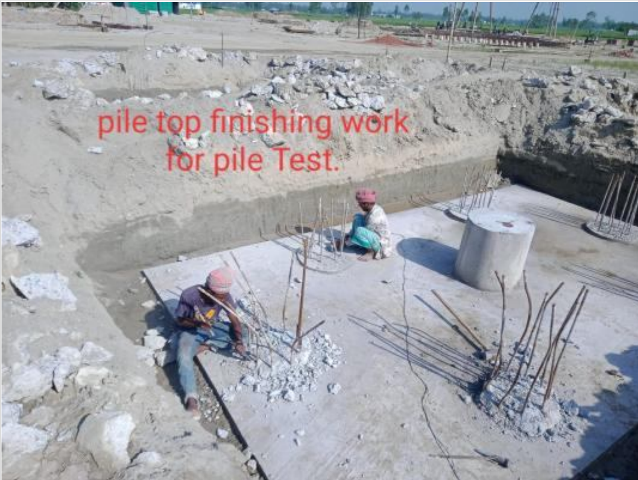
Pile head finishing for test on 07-04-23
