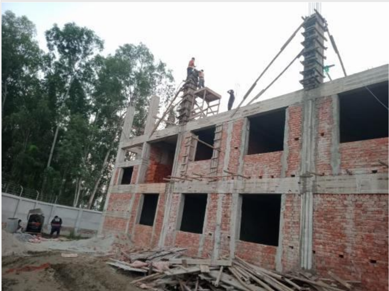
Dorm. Bldg. 2nd floor column work on 03-11-23
