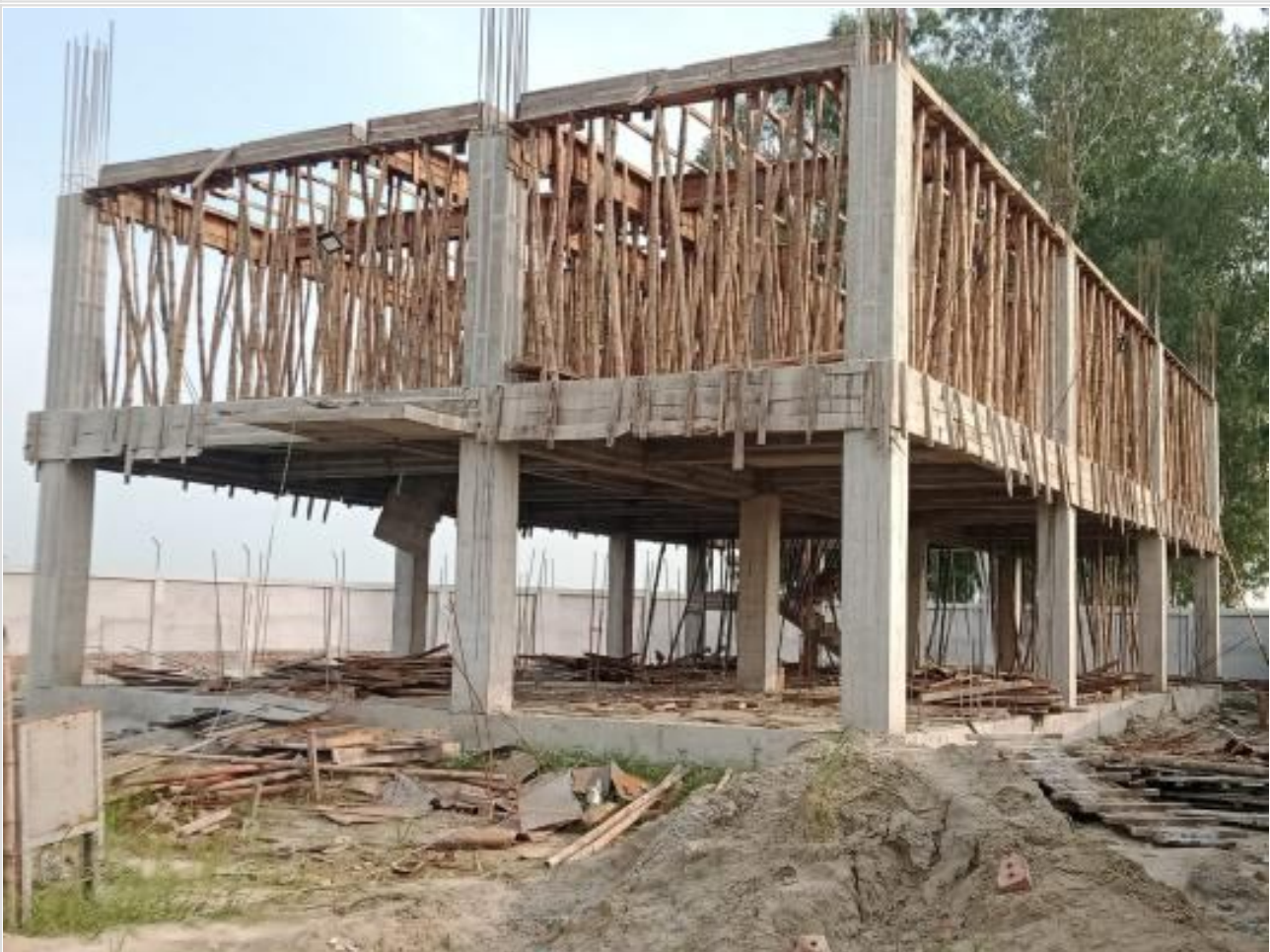
Dorm. Bldg. 2nd floor shuttering work on 03-09-23
