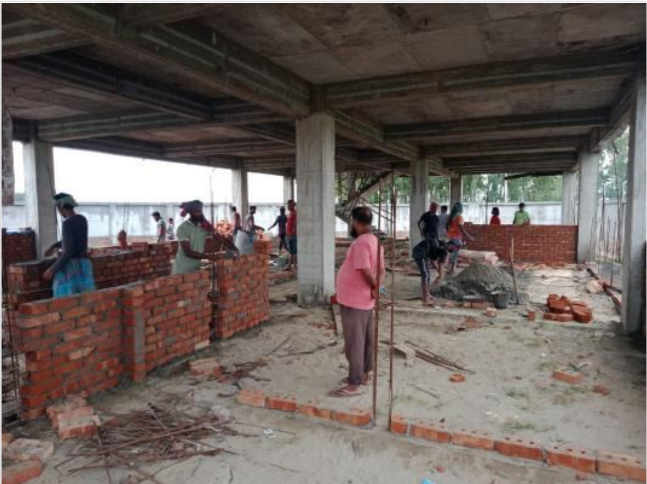
Dorm. Bldg GF Brick work on 22-09-23
