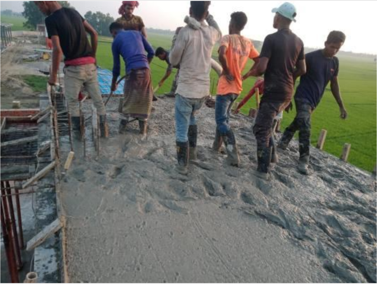
Comp. Bldg. Roof top concreting work on 16-09-23
