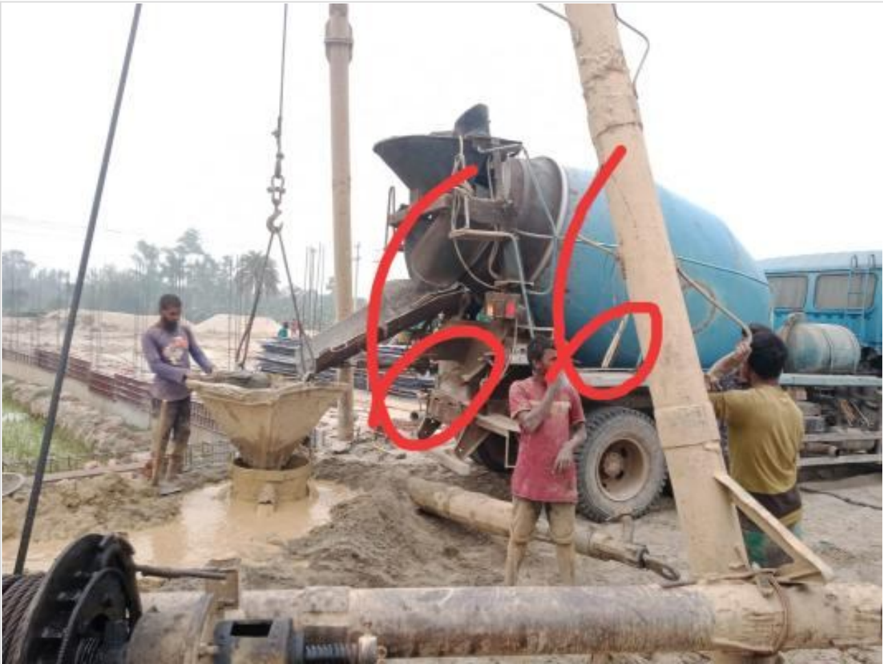
Ready mix concreting of pile on 16-03-23
