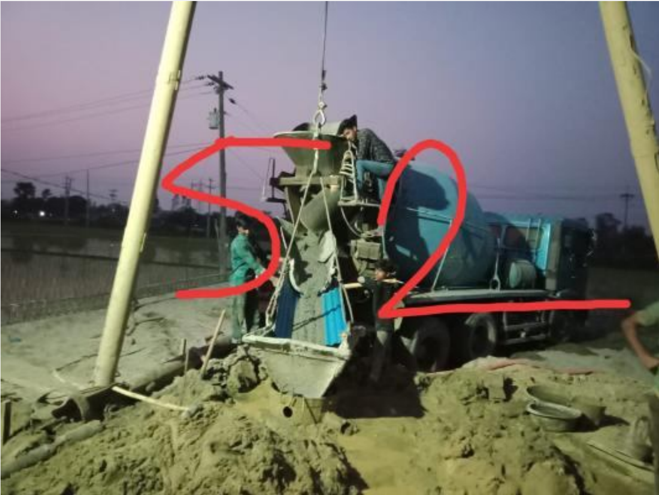
Ready mix concreting of pile on 10-03-23
