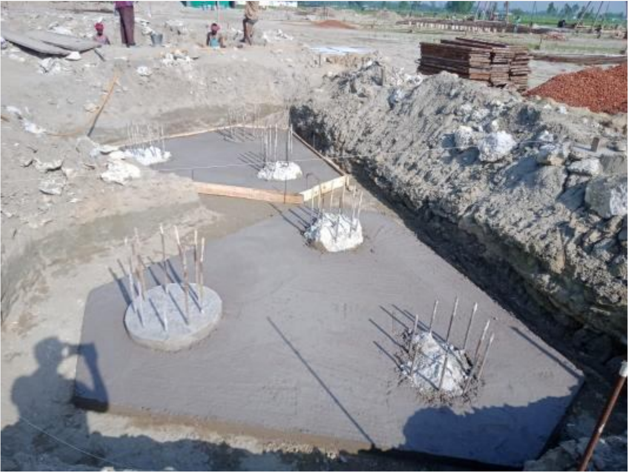
Pile cap CC work on 05-04-23
