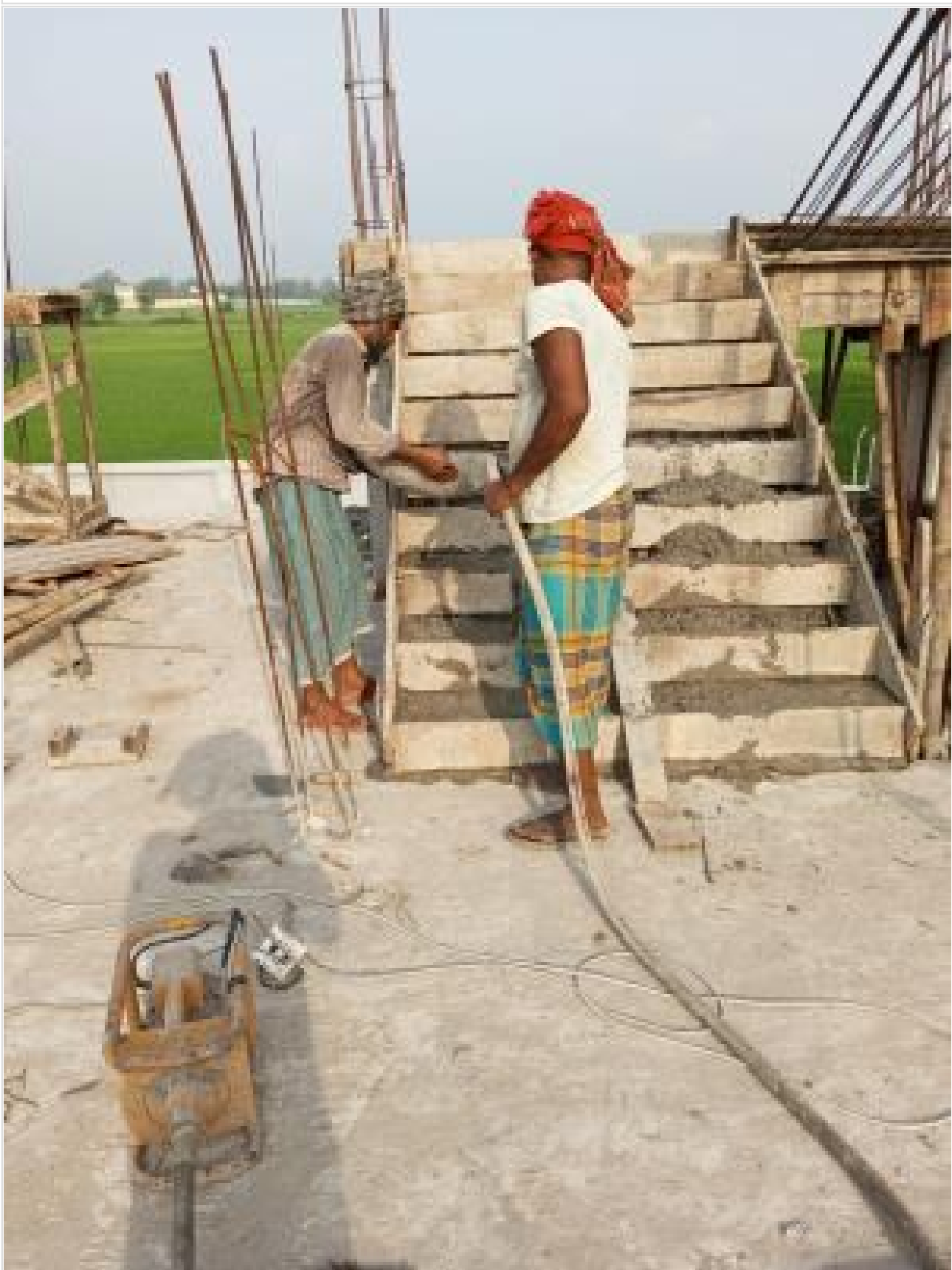
Dorm. Bldg. 1st flight stair casting on 30-08-23
