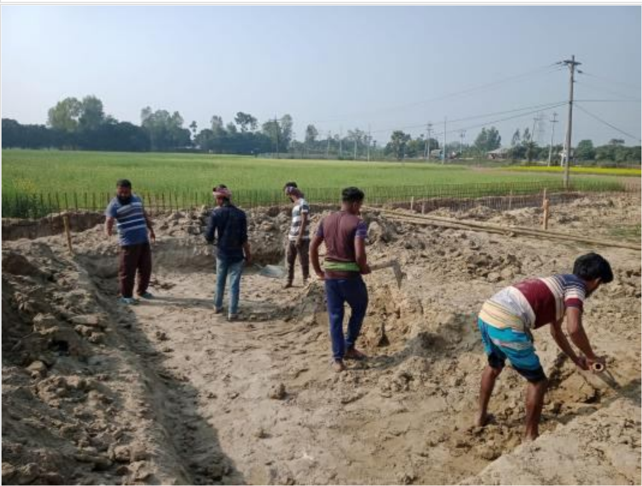
Exaction for Pile mud tank on 02-02-23
