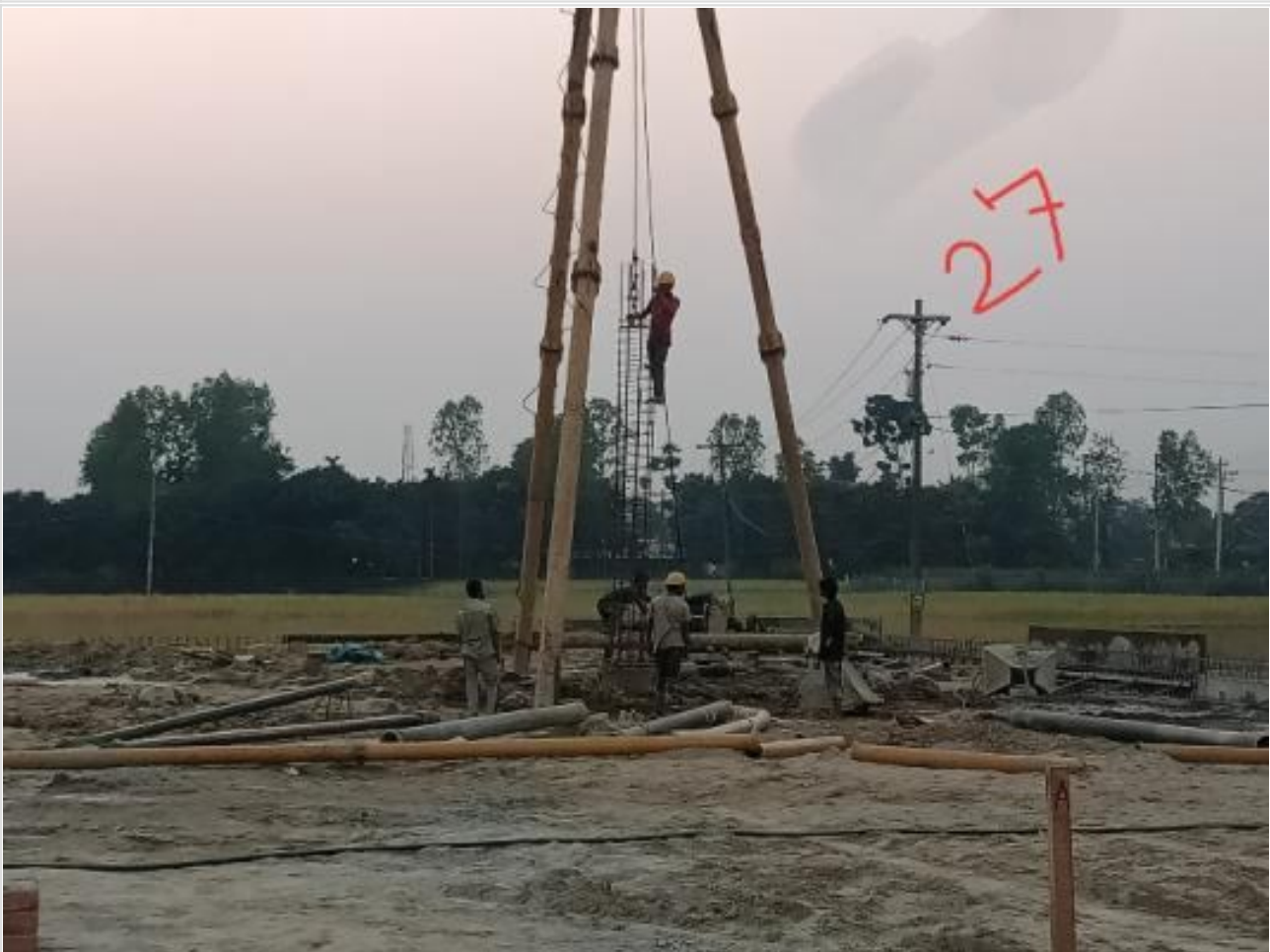
Com. Bldg. 27th pile boring on 25-02-23
