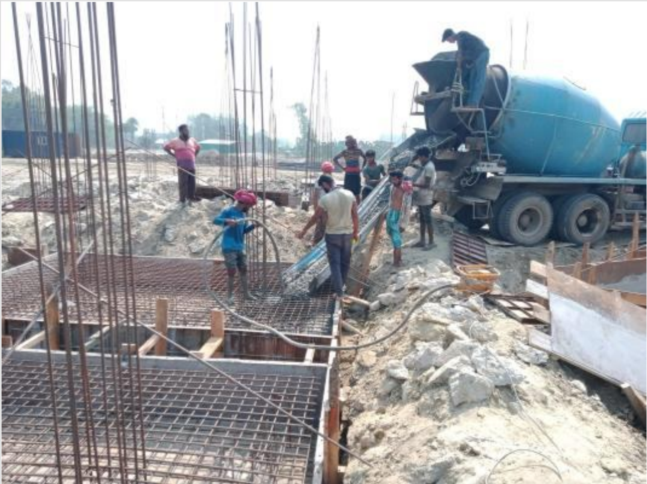
Com. Bldg. Pile cap casting on 17-04-23
