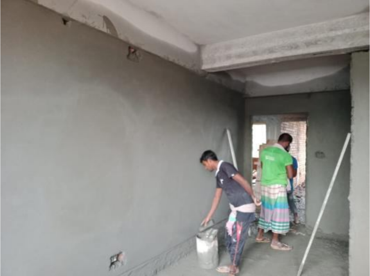
Comp. Bldg. Plaster work on 20-09-23
