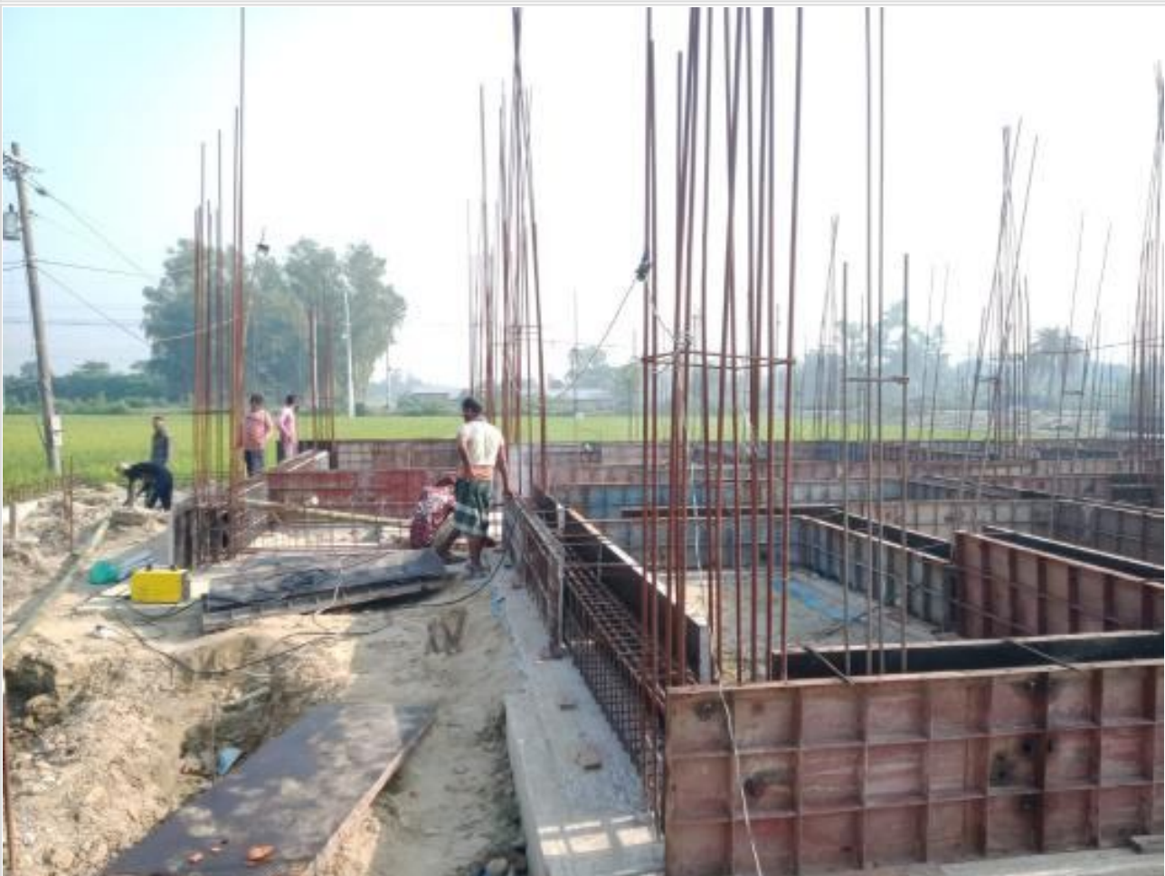
Comp. Bldg. GB Shuttering work on 08-05-23
