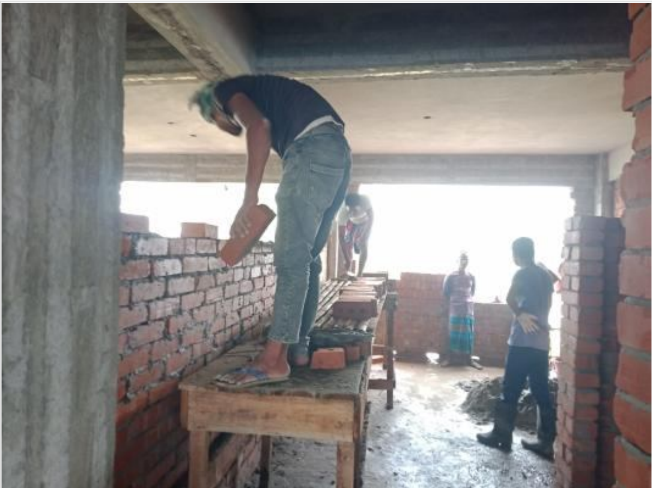
Comp. Bldg. 1st floor brick wall on 04-09-23
