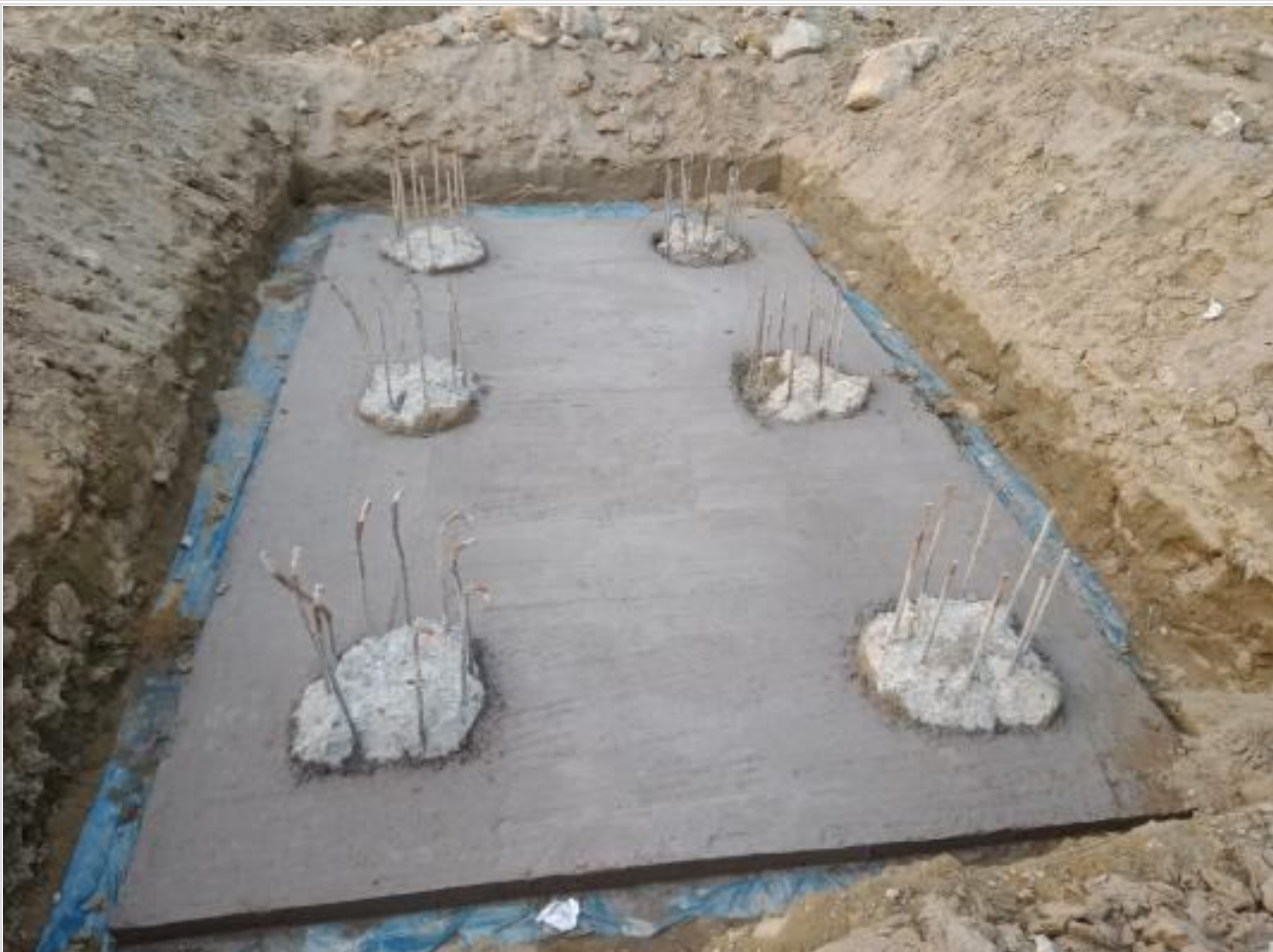
Pile head finishing for test on 03-04-23
