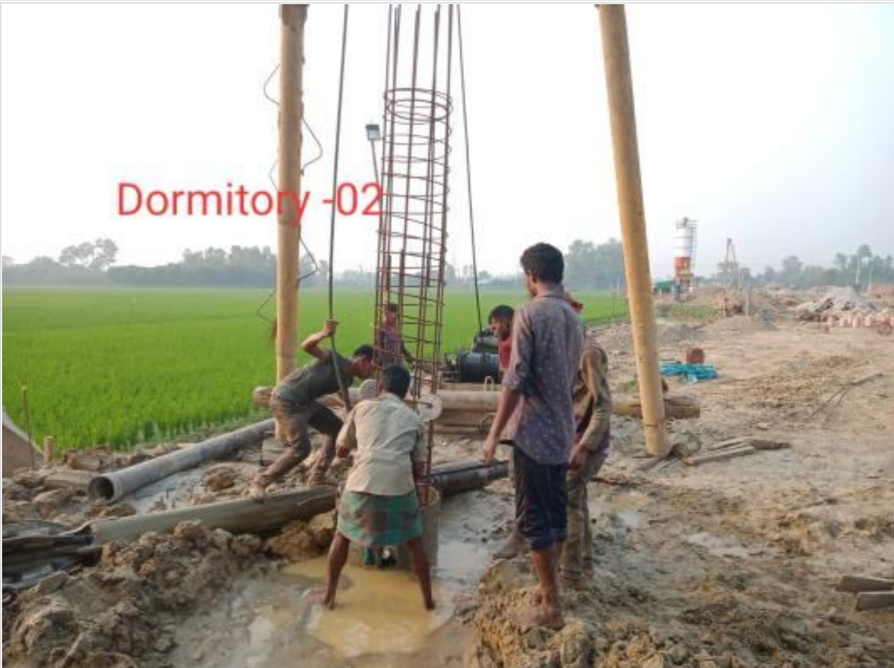
Pile head breaking on 24-03-23
