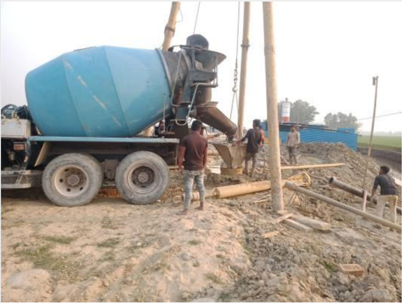
Ready mix concreting of pile on 16-02-23
