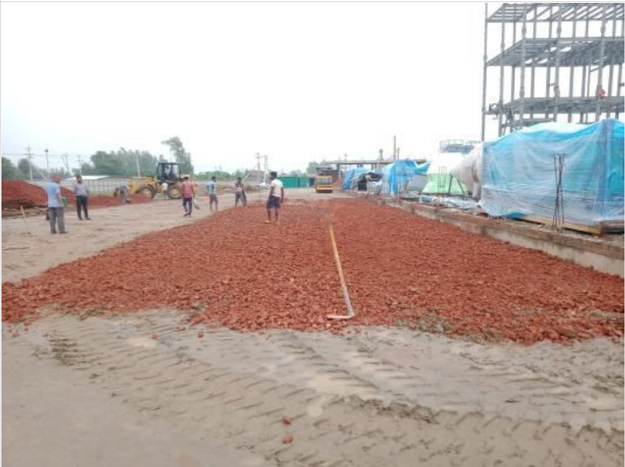
Road work on 24-08-23
