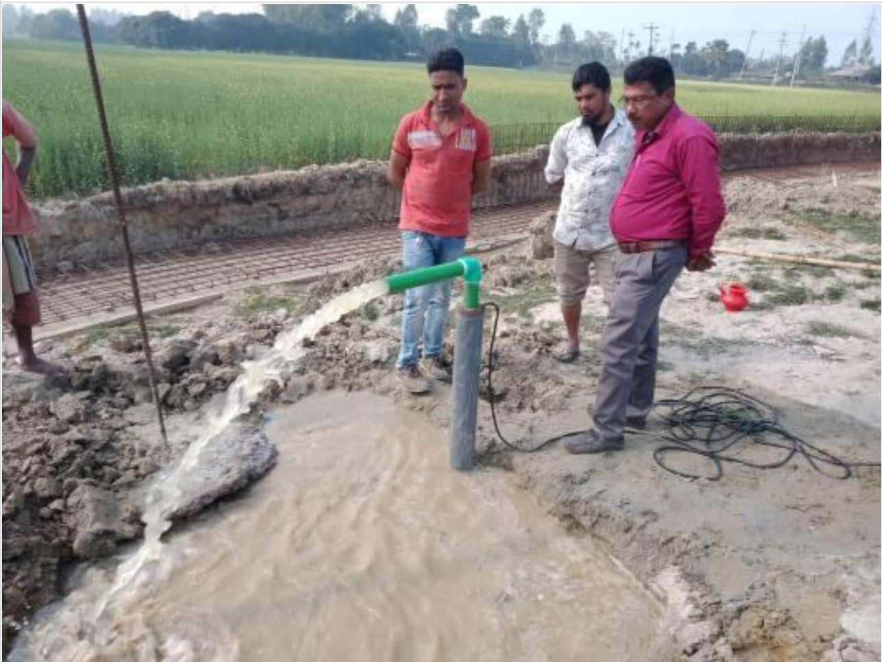
Deep tube well sinking on 01-02-23
