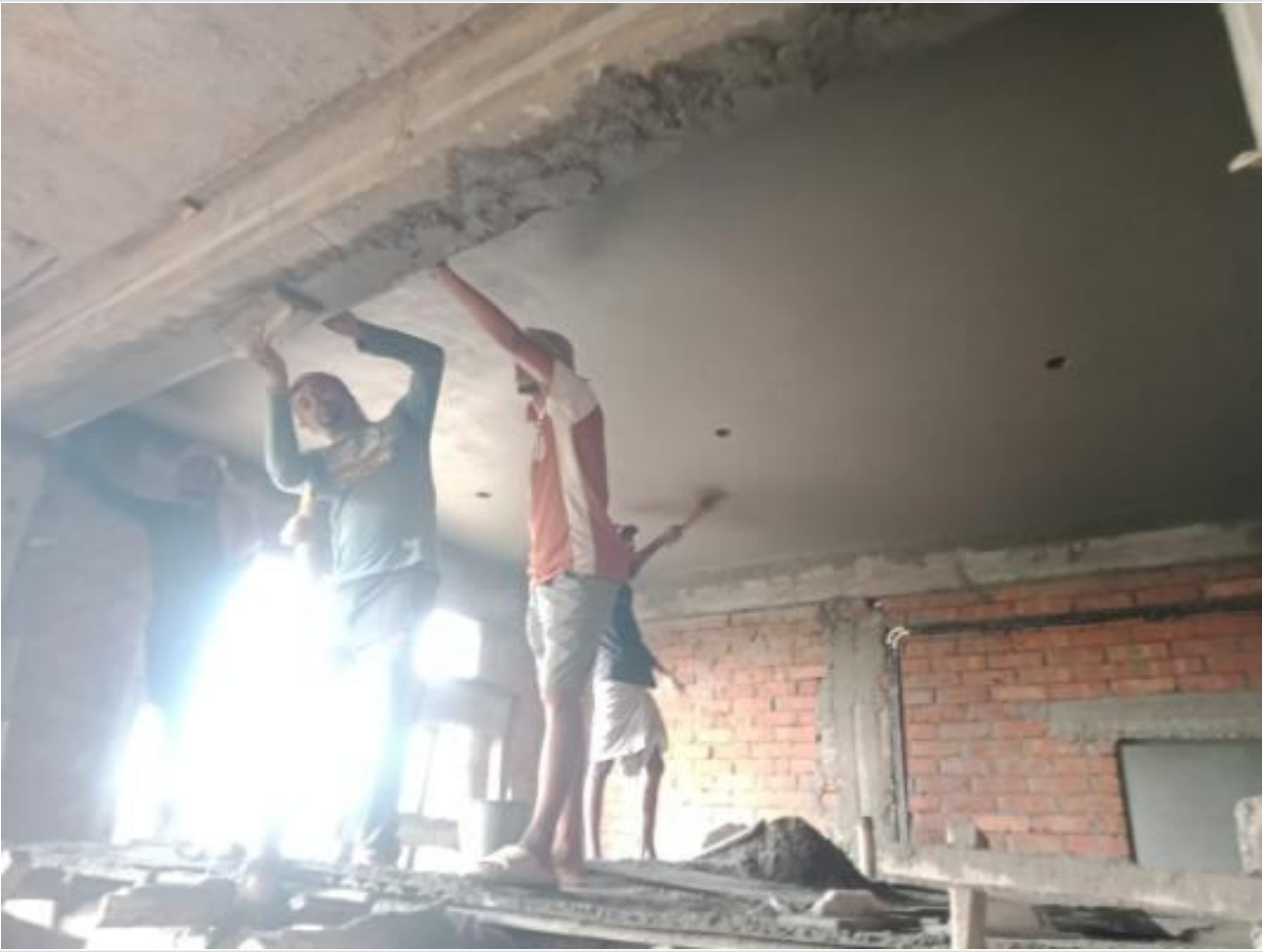
Ceiling plaster on 25-10-23
