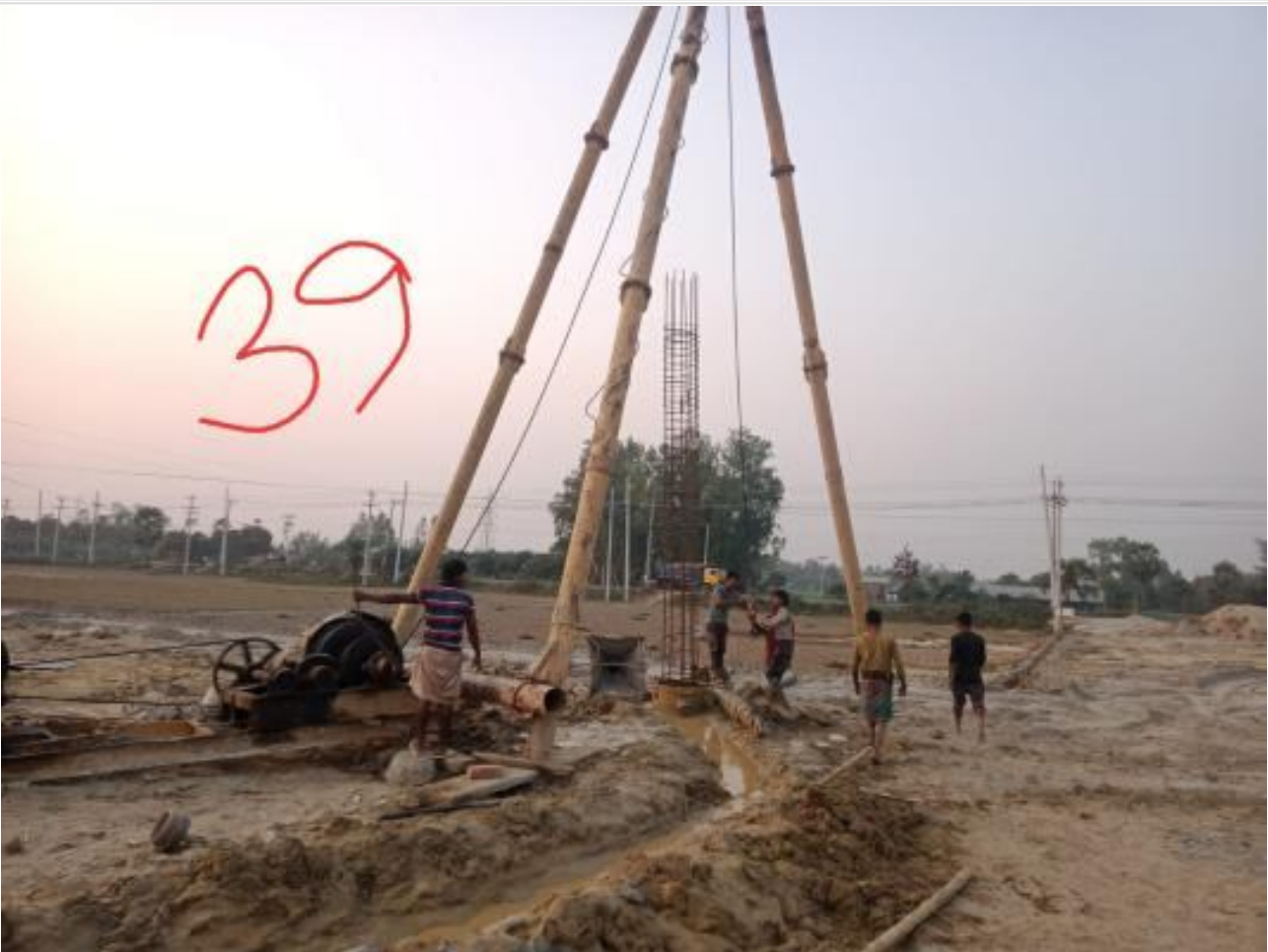
Com. Bldg. 39 pile boring on 02-03-23
