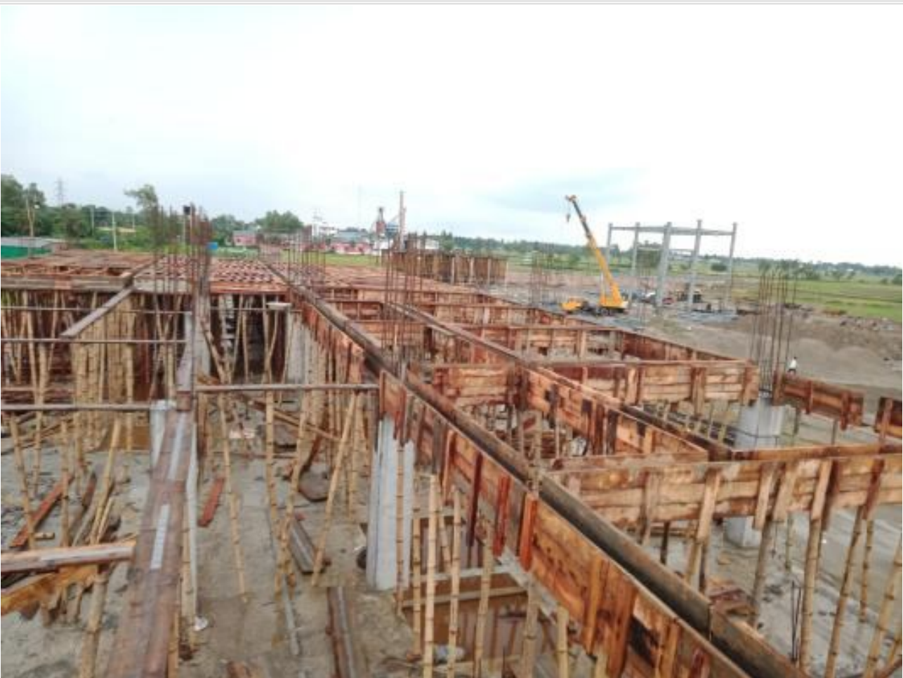
Comp. Bldg. 2nd Floor Slab beam shuttering on 21-07-23
