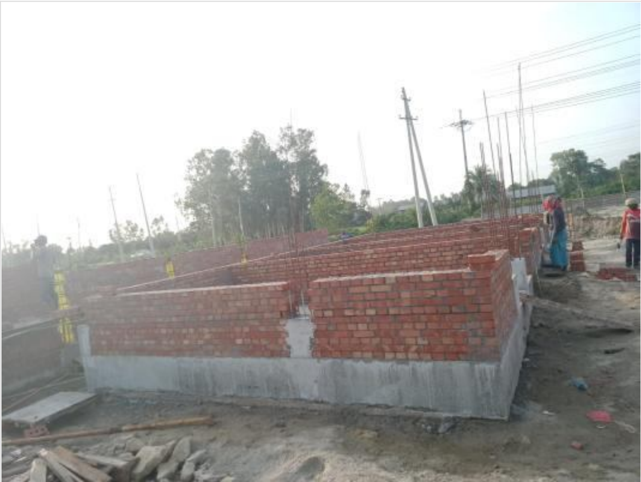
Gate house Brick work on 01-06-23
