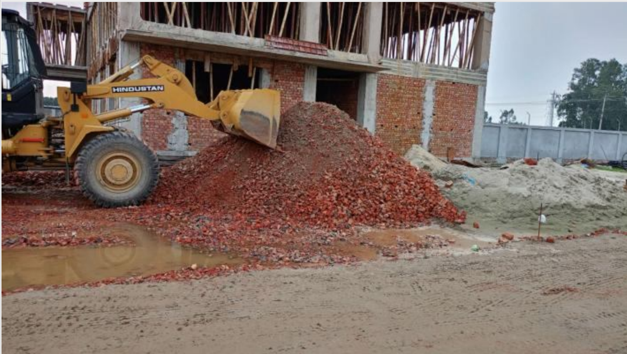
Sub-base-Khoa unloading on 14-08-23
