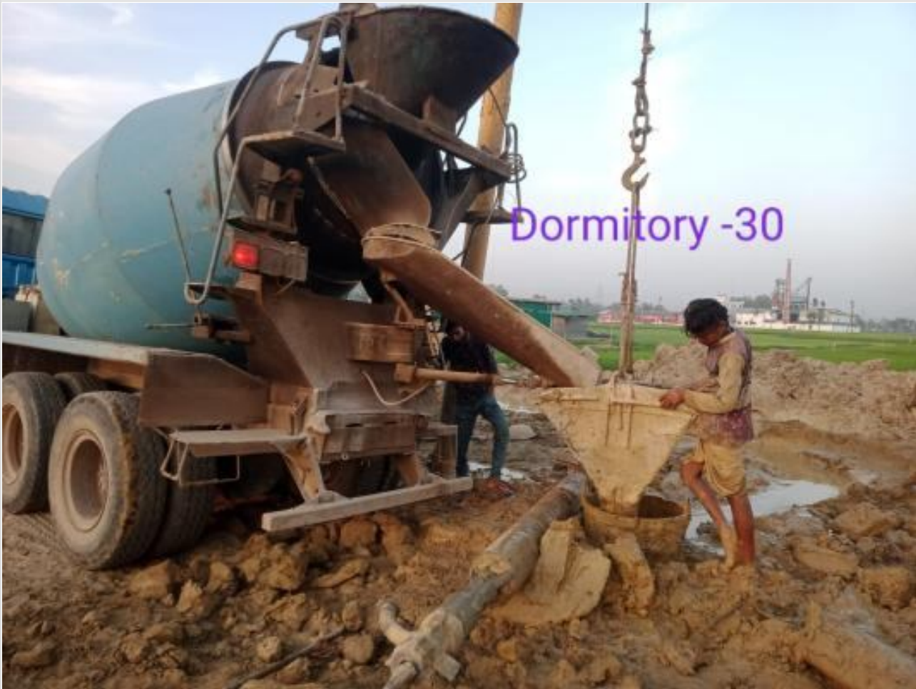
Ready mix concreting of pile on 08-04-23
