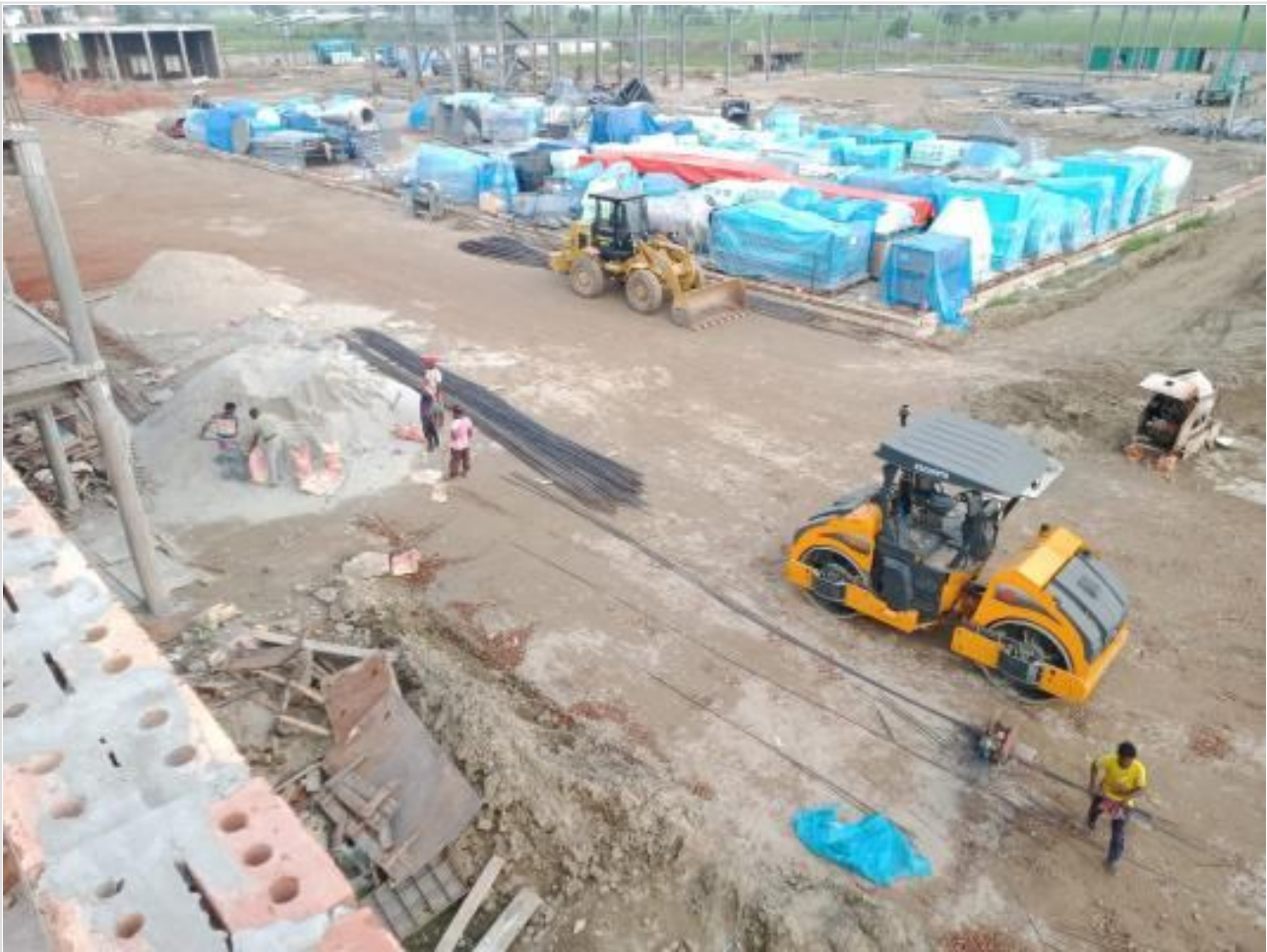
Road work on 03-09-23
