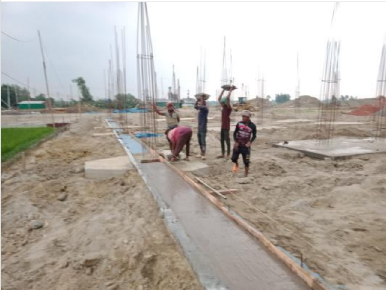
Comp. Bldg. C.C concreting on 29-04-23
