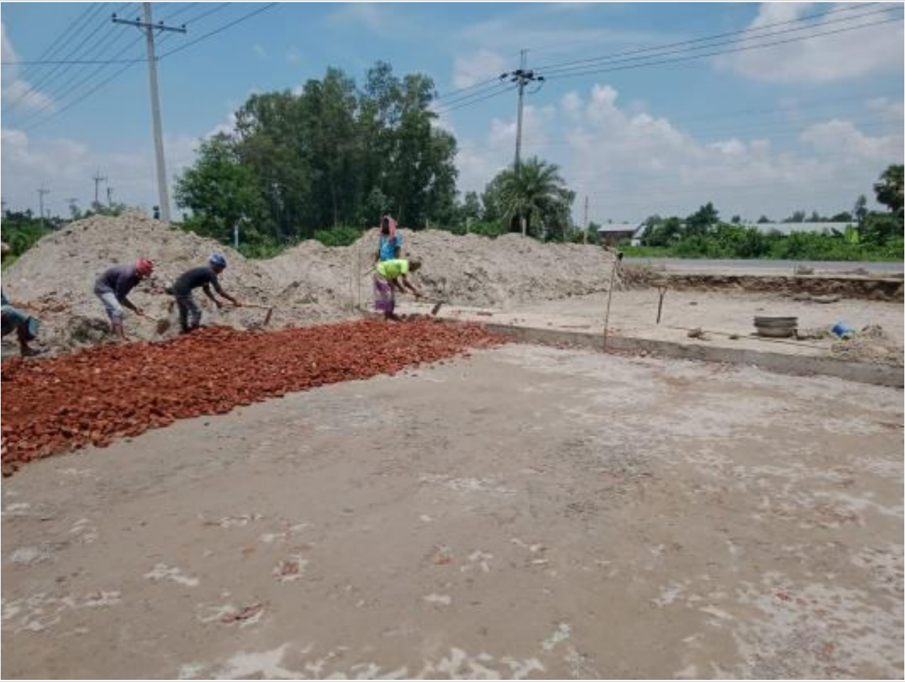
Road work on 31-07-23
