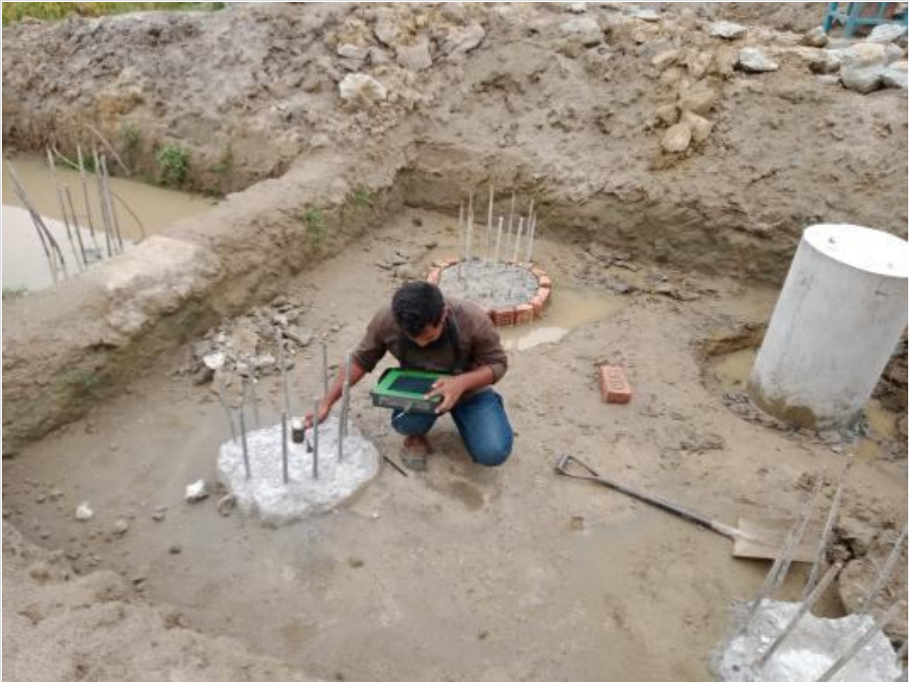
Pile integrity test on 19-05-23
