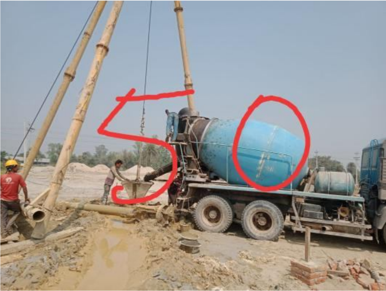
Ready mix concreting of pile on 09-03-23
