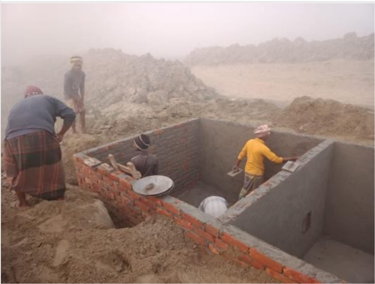
Mud Tank-2 Completed on 12-02-23
