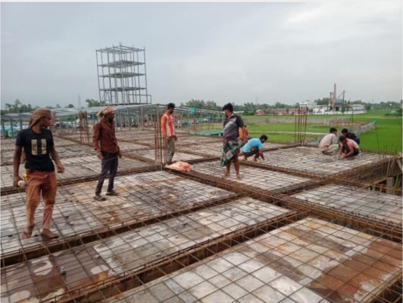
Dorm. Bldg. 2nd floor rebar work on 08-09-23
