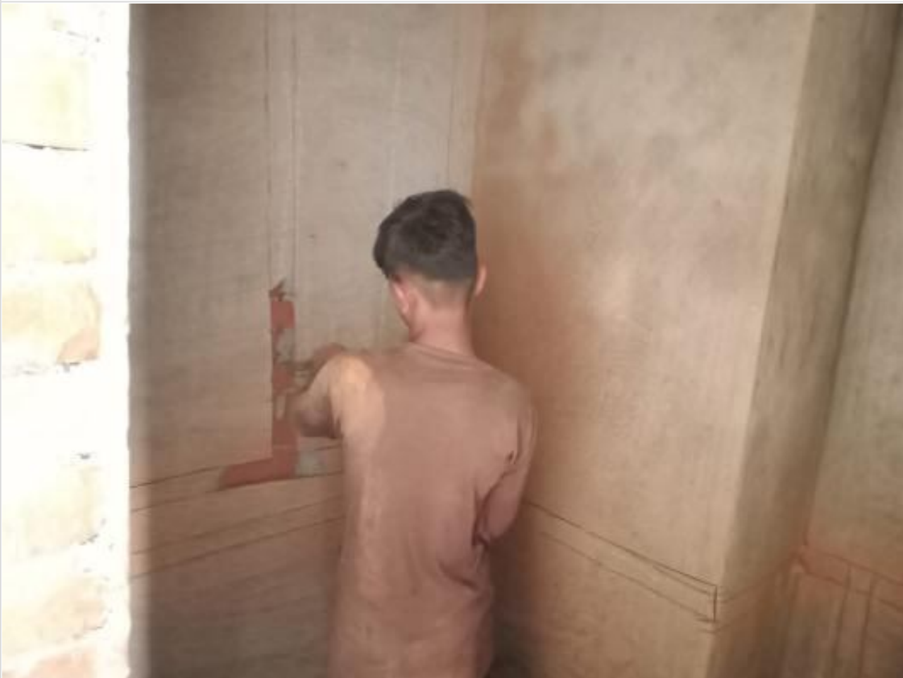
Sanitary group cutting on 06-11-23
