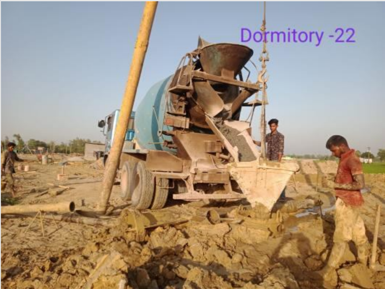
Dorm. Bldg. 22nd pile casting on 06-04-23
