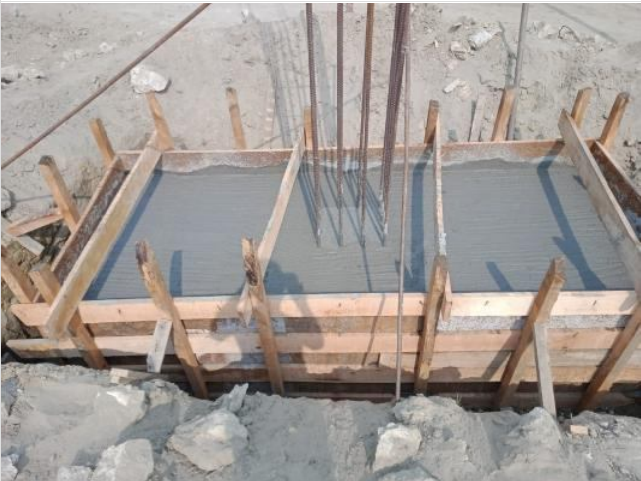
Pile Cap concreting. on 16-04-23
