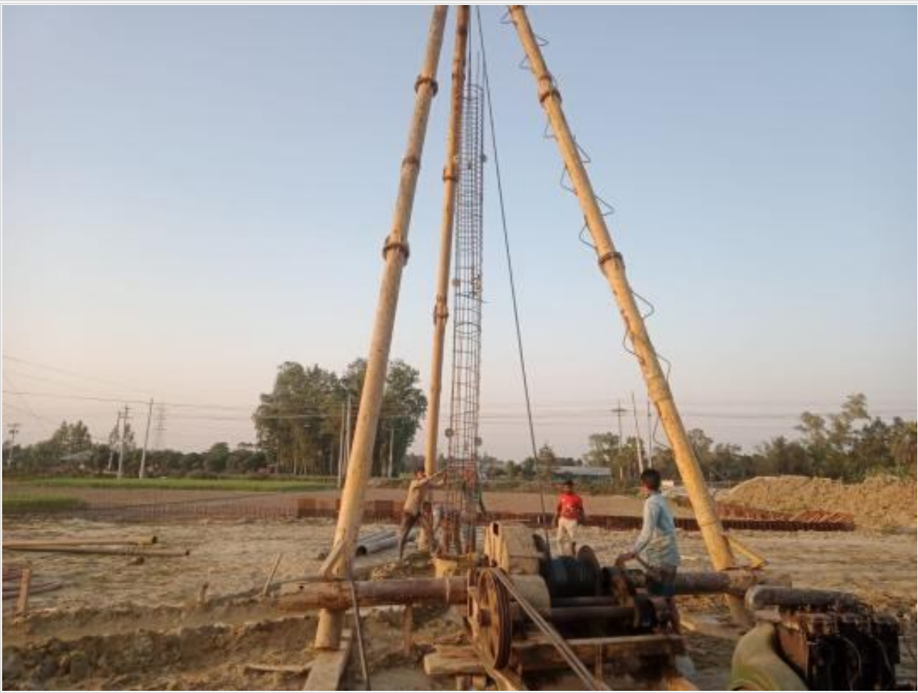
Pile boring work on 13-02-23
