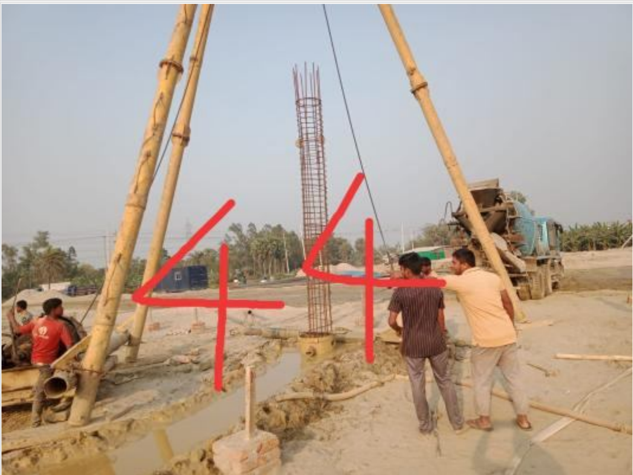
Com. Bldg. 44 pile boring on 05-03-23
