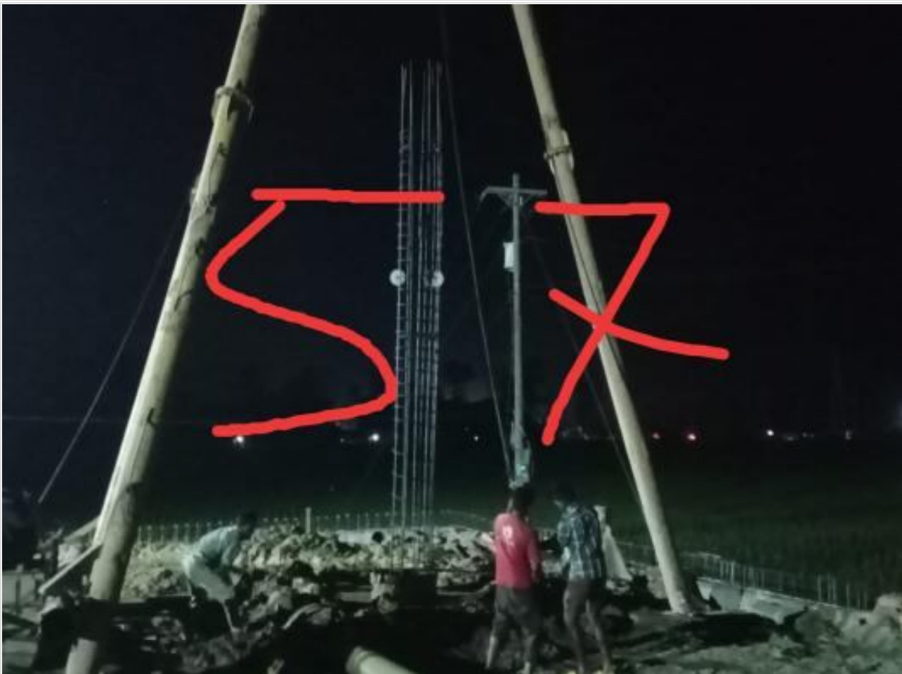
Ready mix concreting of pile on 11-03-23
