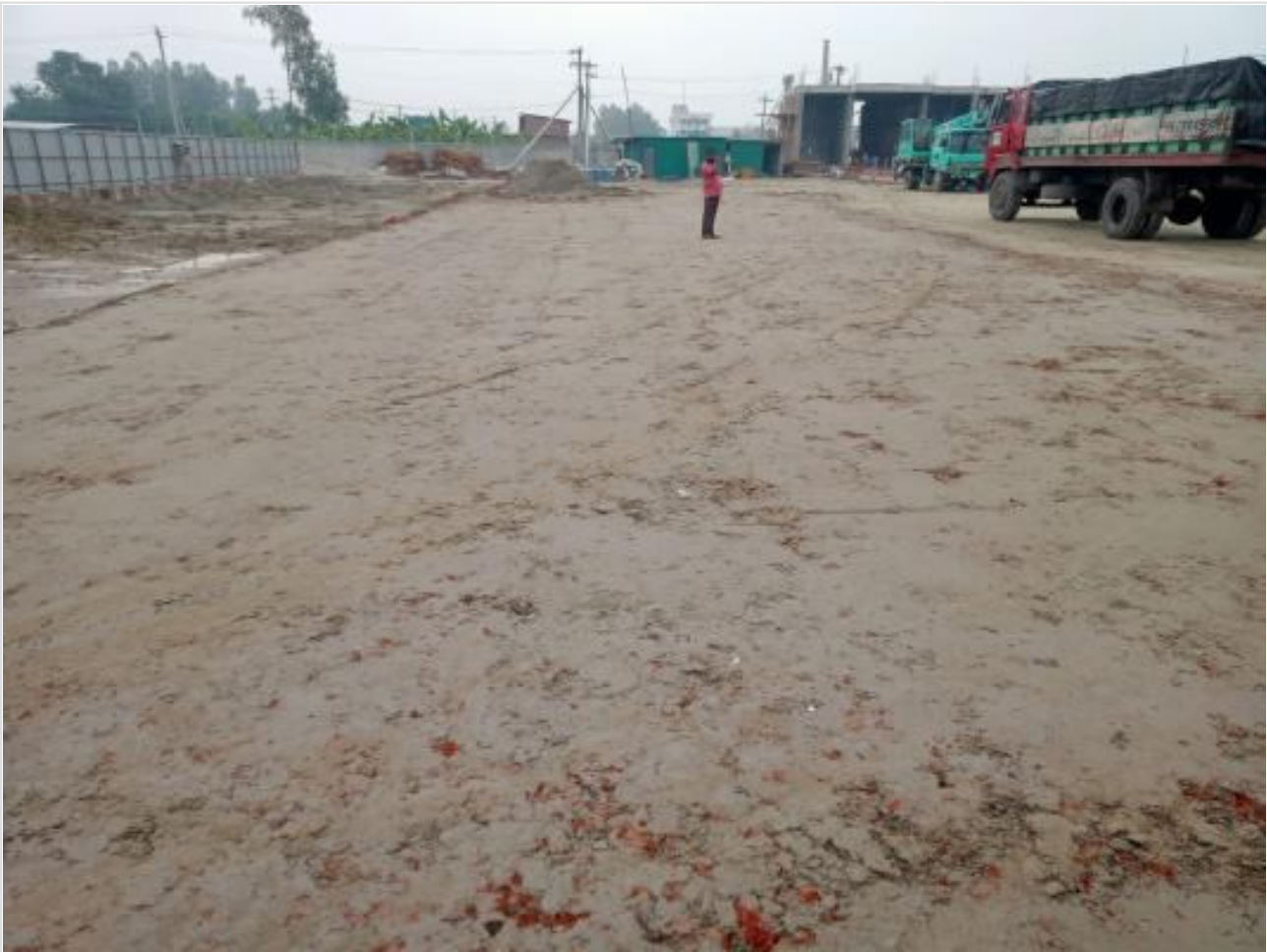
Road work on 13-09-23
