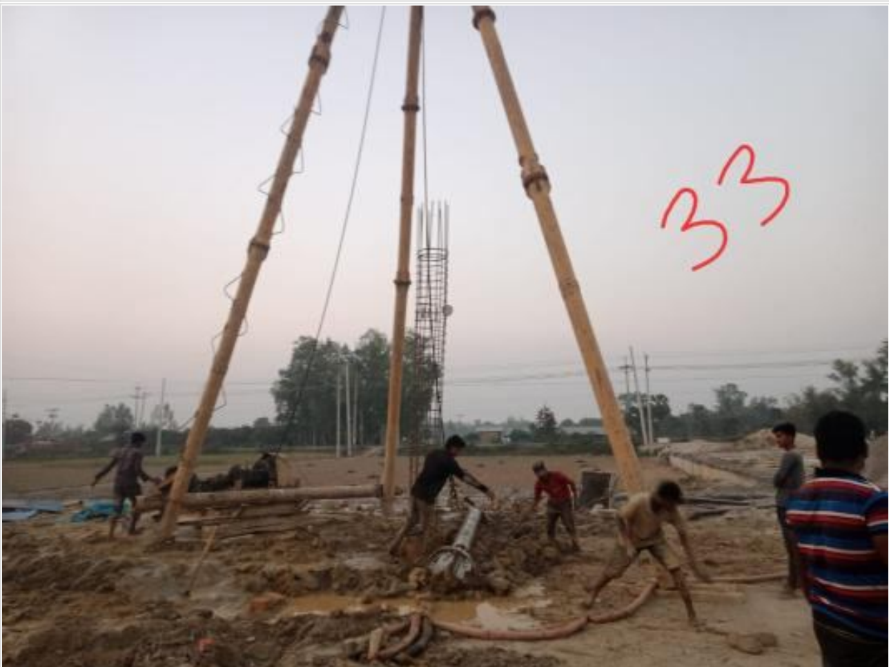
Com. Bldg. 33 pile boring on 27-02-23
