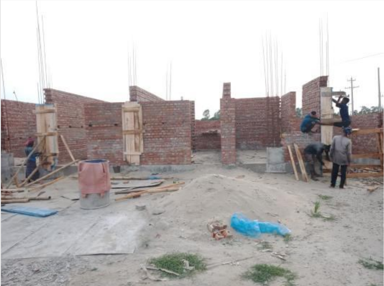
Gate house column shuttering work on 16-06-23
