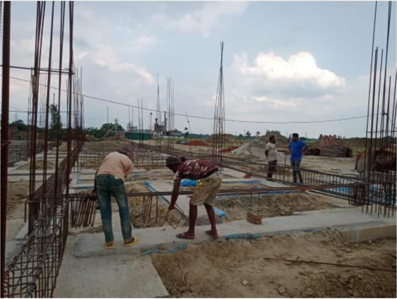
GB Re-bar work on 04-05-23
