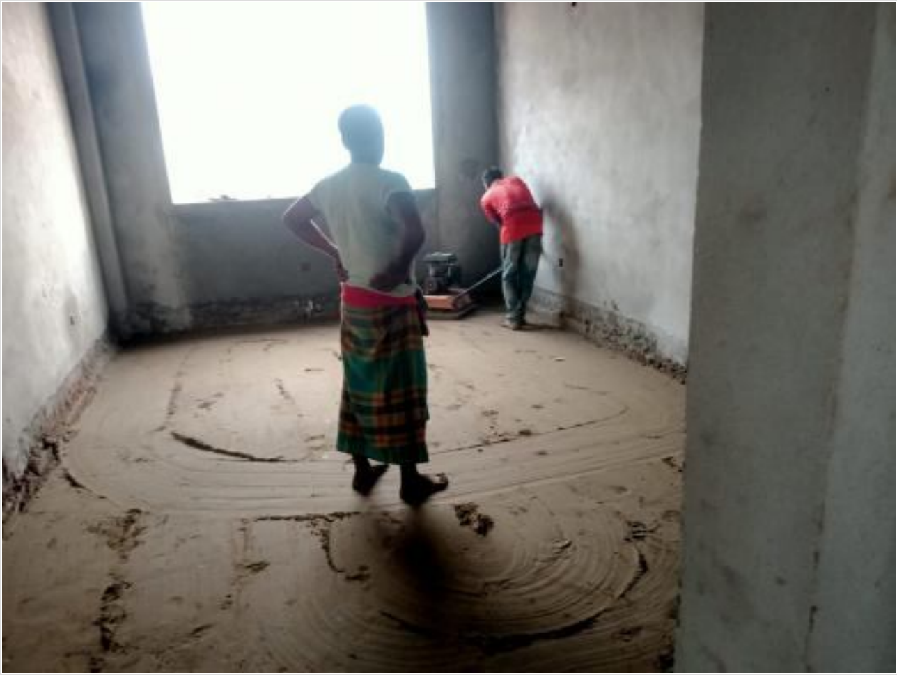
Comp. Bldg floor GF compaction on 11-09-23
