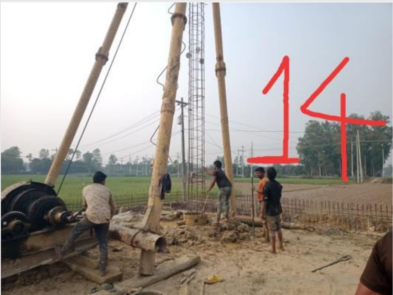
Com. Bldg. 14th pile boring on 18-02-23
