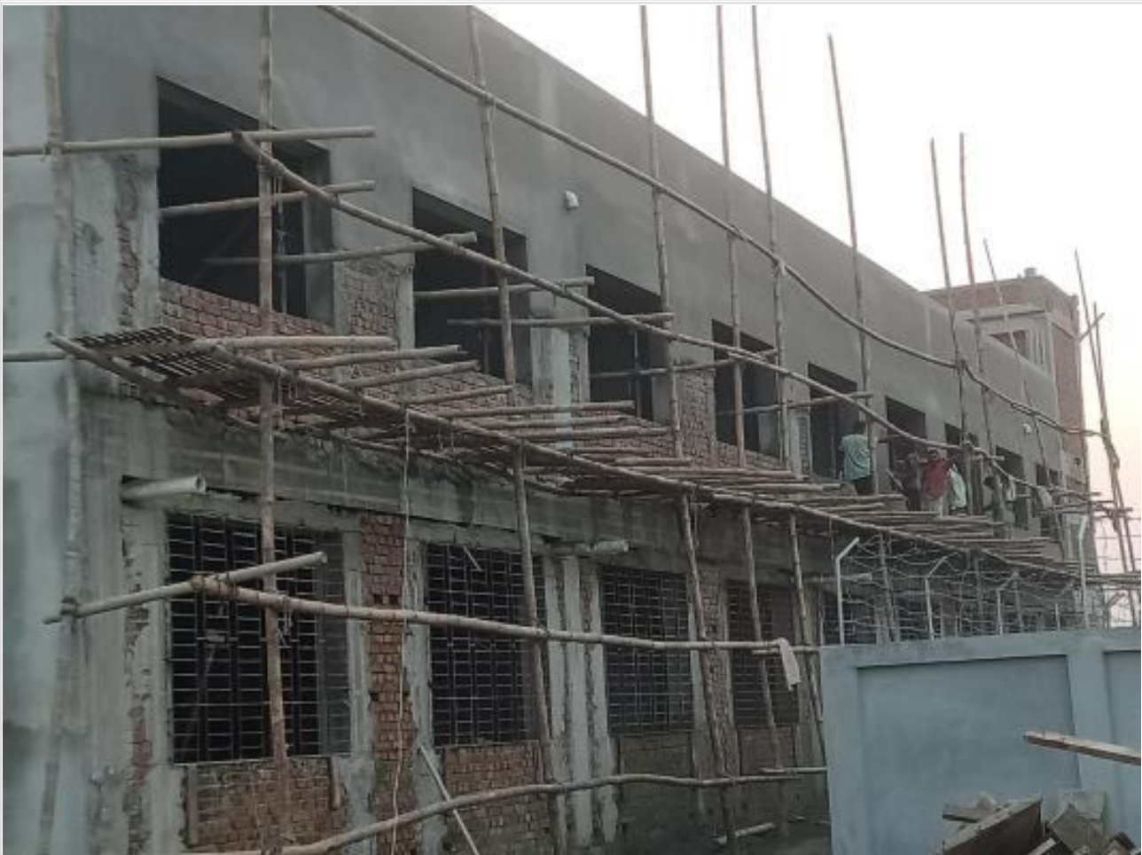
Comp. Bldg. Outside plaster work on 18-10-23
