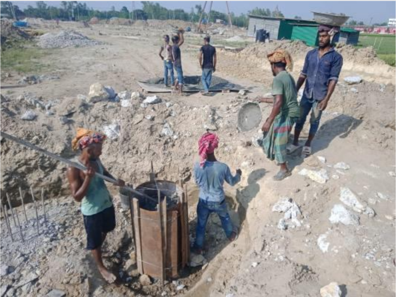
Pile head finishing for test on 09-05-23
