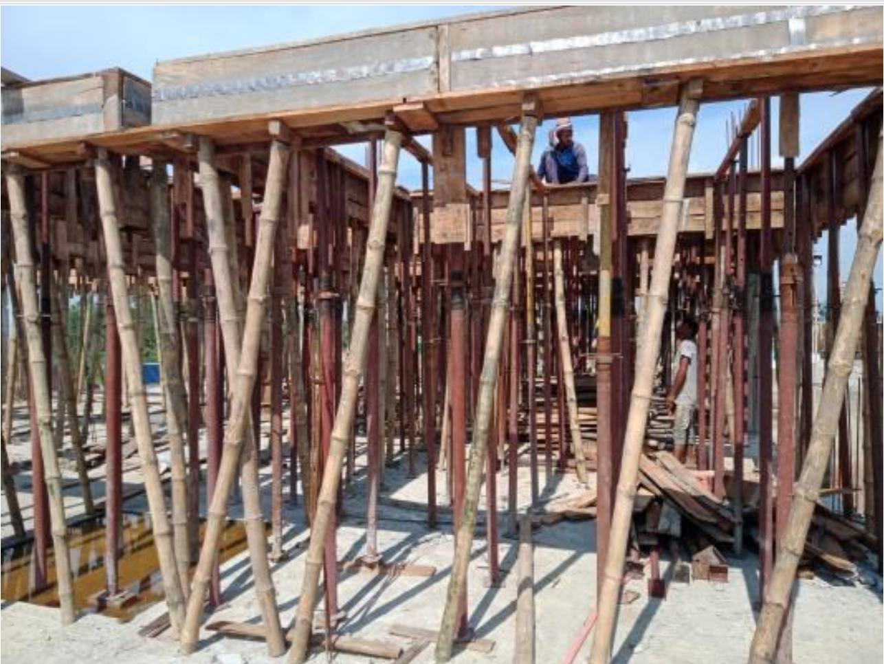
Comp. Bldg. 2nd Floor Slab beam shutteri on 18-07-23
