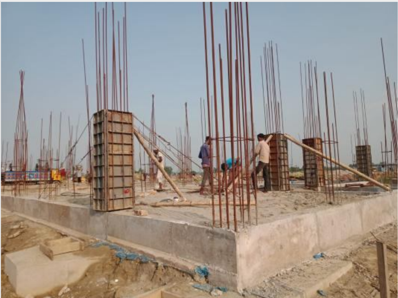
Comp. Bldg. Column shuttering on 24-05-23
