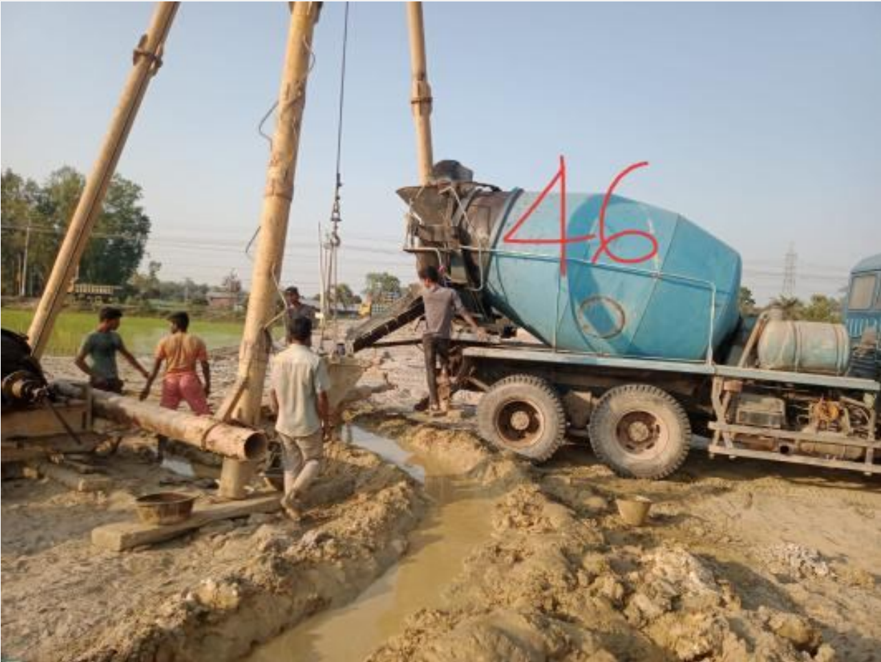
Ready mix concreting of pile on 07-03-23
