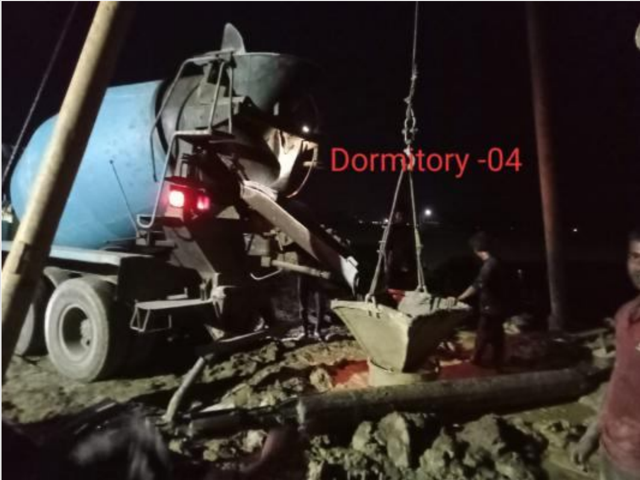
Ready mix concreting of pile on 26-03-23
