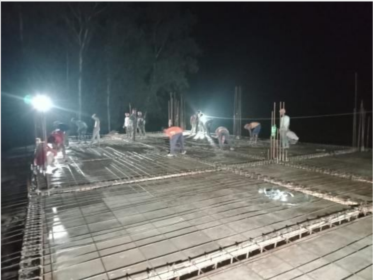
Dormitory 1st Floor Re-bar work on 06-08-23
