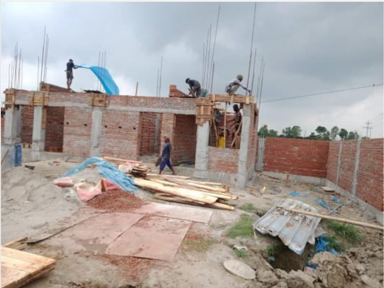
Gate House Lintel casting on 23-06-23
