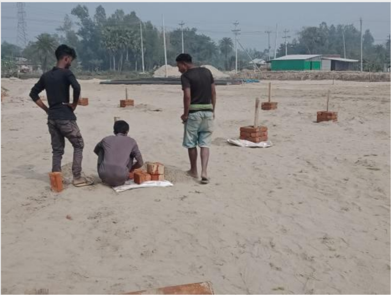
Brick-work around Pile point on 05-02-23
