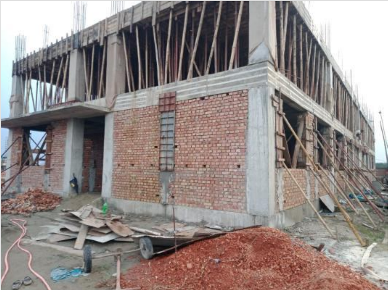
Comp.Bldg.GF Brick work on 09-08-23
