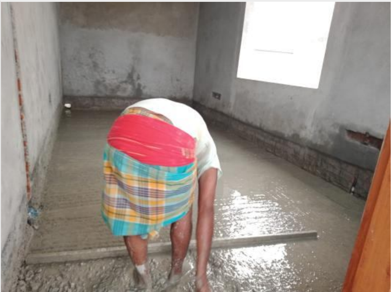
Gate House floor casting on 01-09-23
