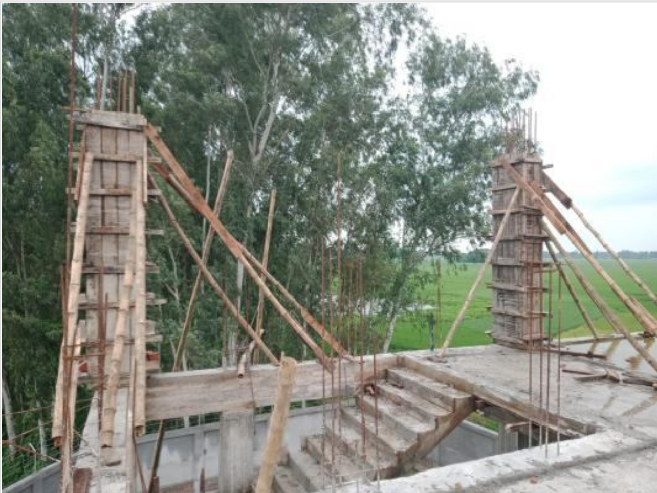
Dorm. Stair room column shuttering on 04-10-23
