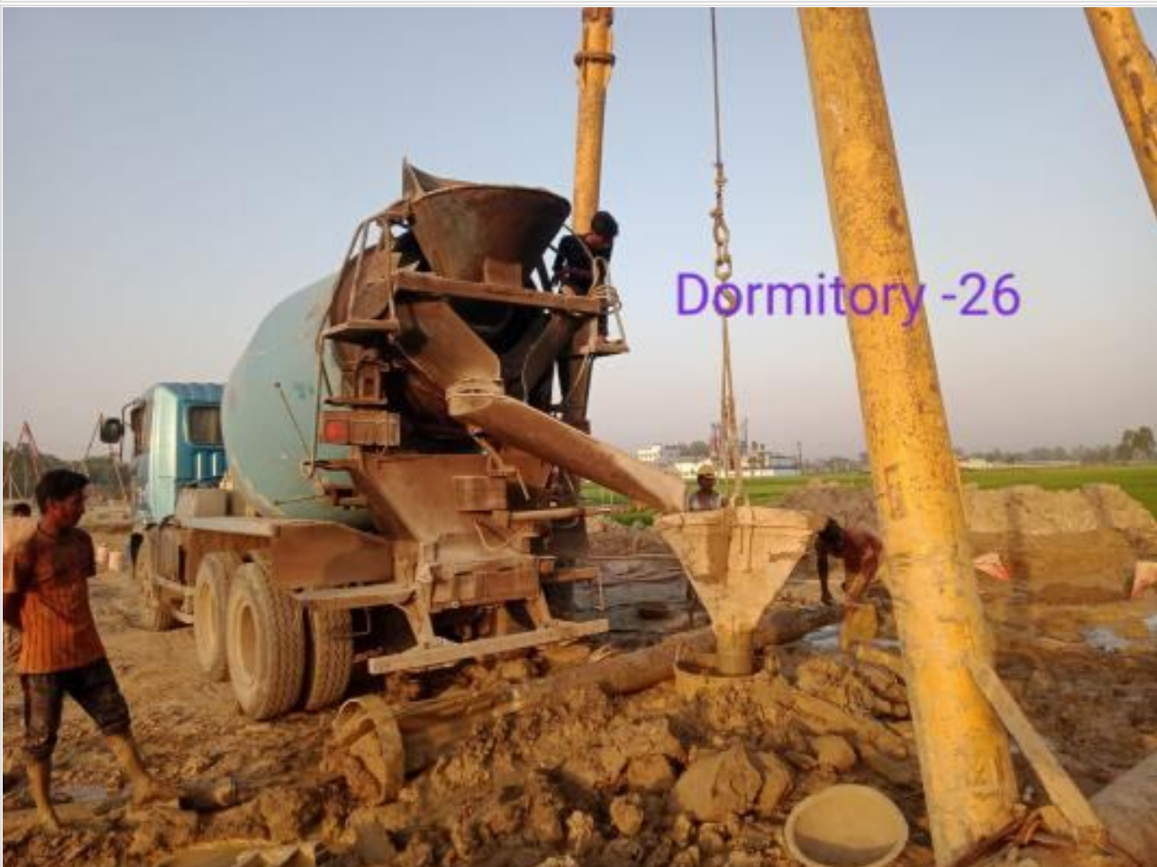
Dorm. Bldg. 22nd pile casting on 06-04-23
