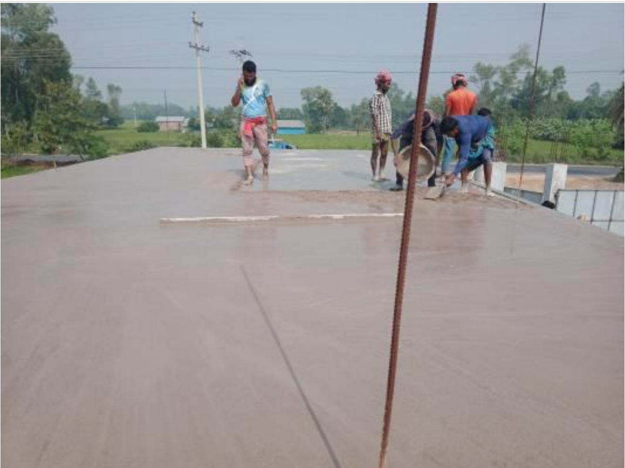
Gate roof top water proofing casting on 08-11-23
