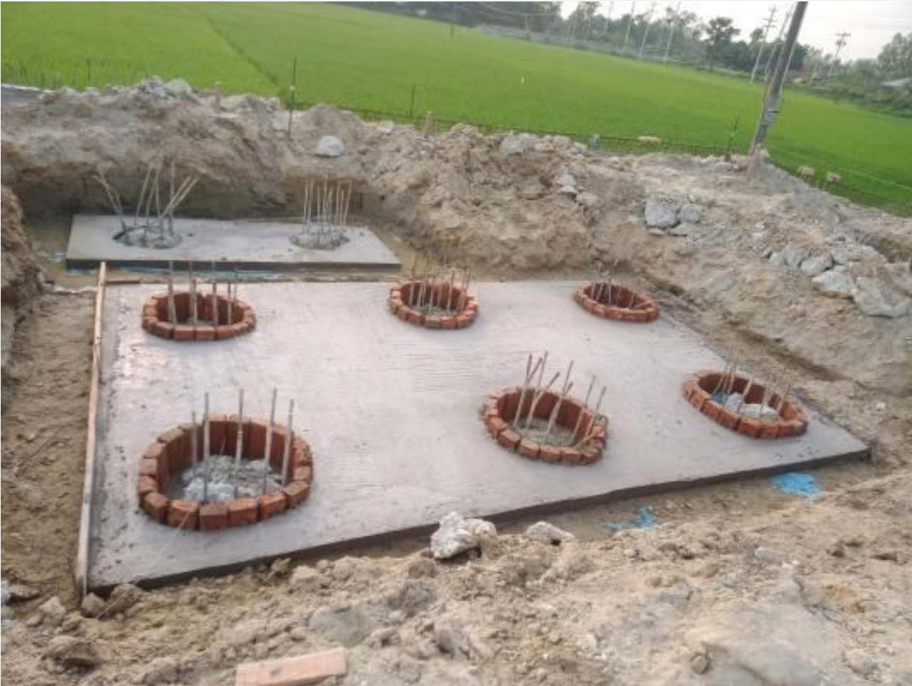
Pile cap bottom cc casting. on 04-04-23
