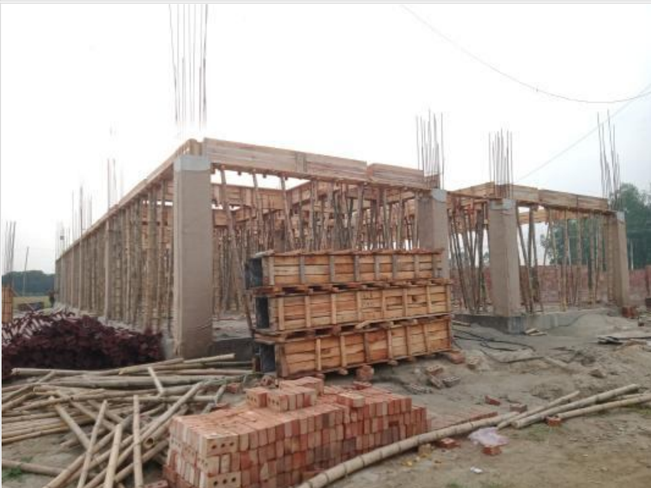
Comp. Bldg. Slab beam shuttering on 07-06-23
