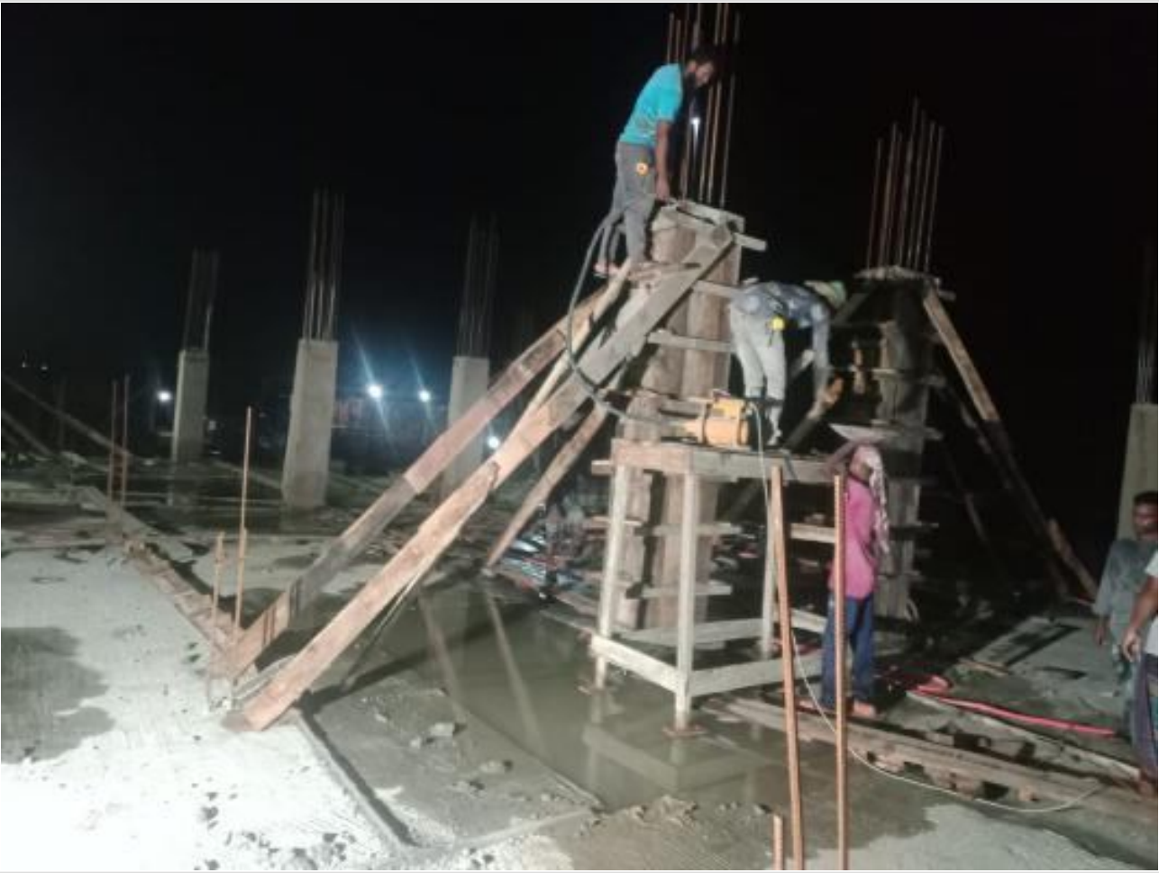
Comp. Bldg 1st floor column casting on 13-07-23
