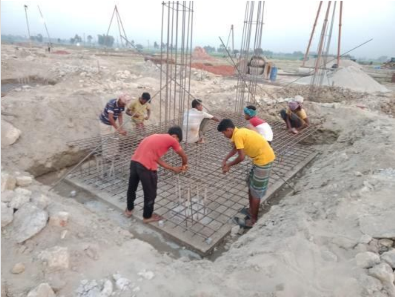
Com. Bldg. Pile cap work on 10-04-23
