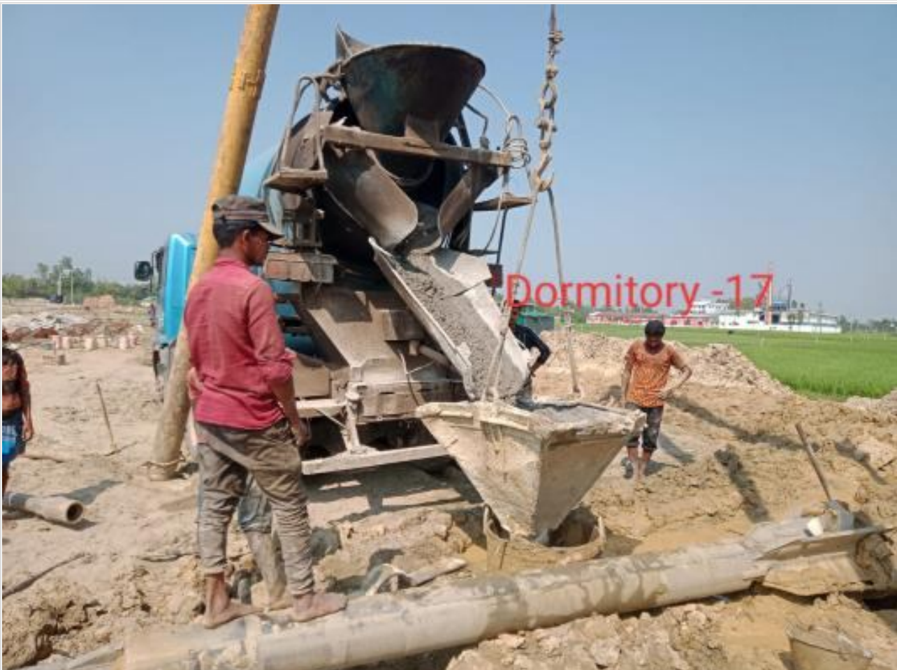
Ready mix concreting of pile on 02-04-23
