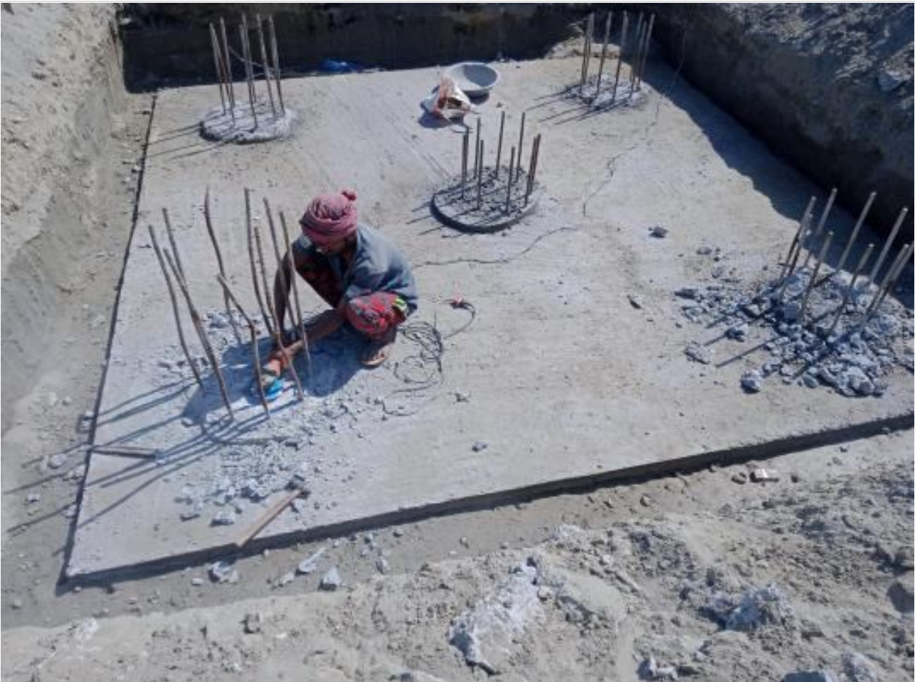
Pile cap CC work on 05-04-23
