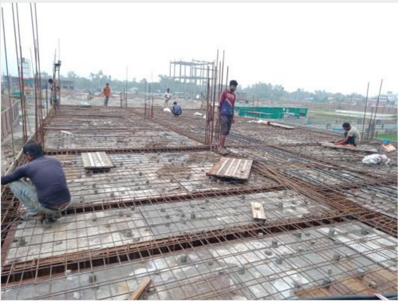
Dormitory Slab Electric Pipe Laying on 09-08-23
