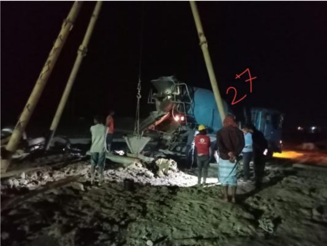
Ready mix concreting of pile on 25-02-23
