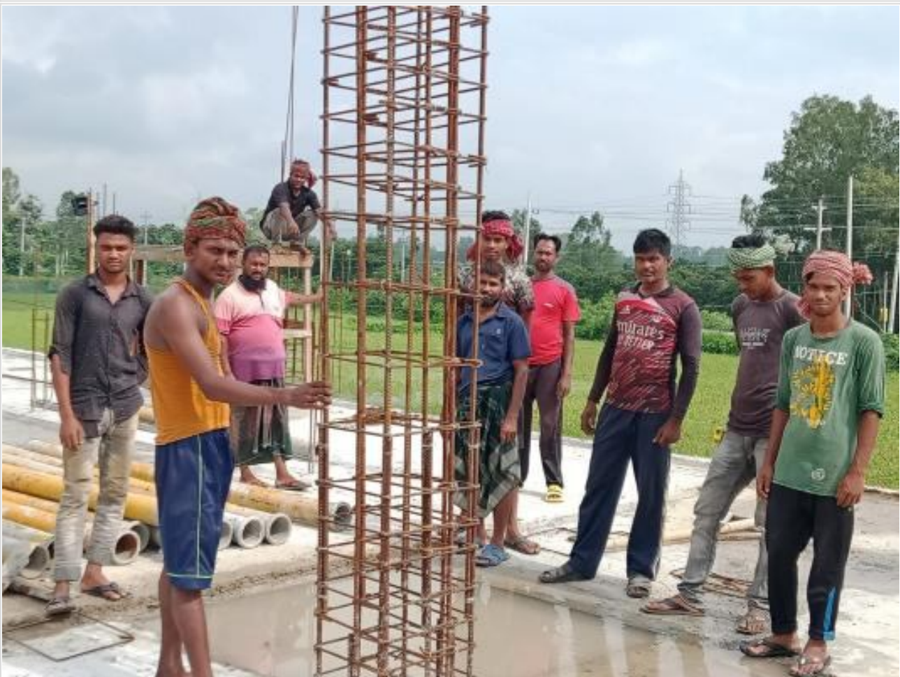
Civil Manpower on 08-07-23
