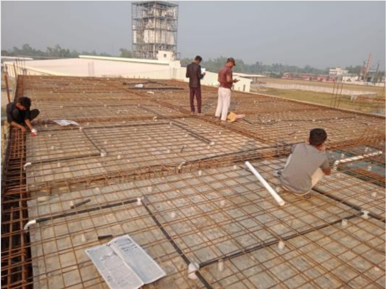
Dormitory-3rd Floor Slab Electrical Pipe on 18-12-23
