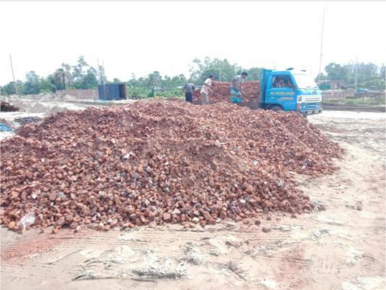
Materials arrive at site for road on 19-07-23
