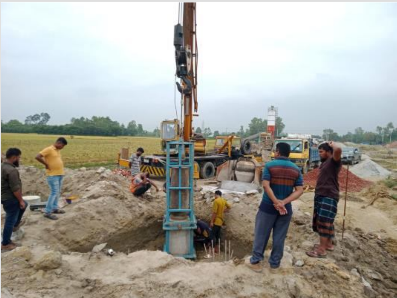
Pile load test on 19-05-23
