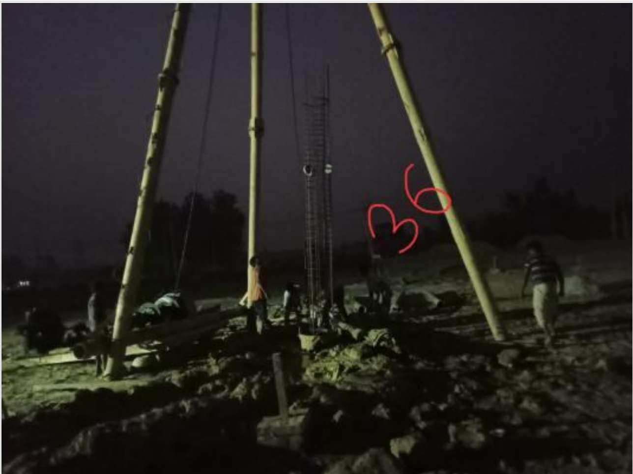
Com. Bldg. 36 Pile Boring on 28-02-23
