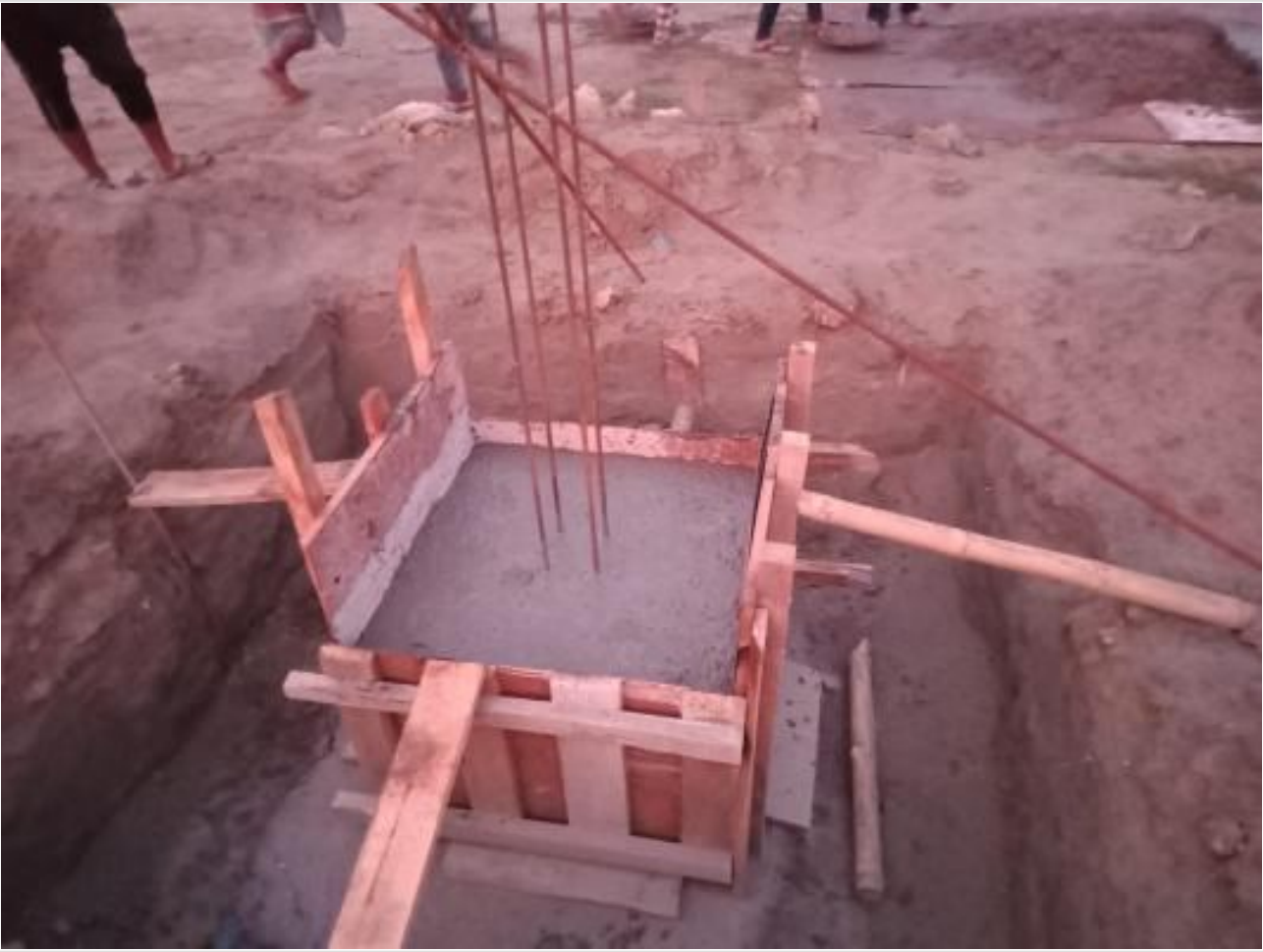
Gate house pile cap casting on 12-05-23
