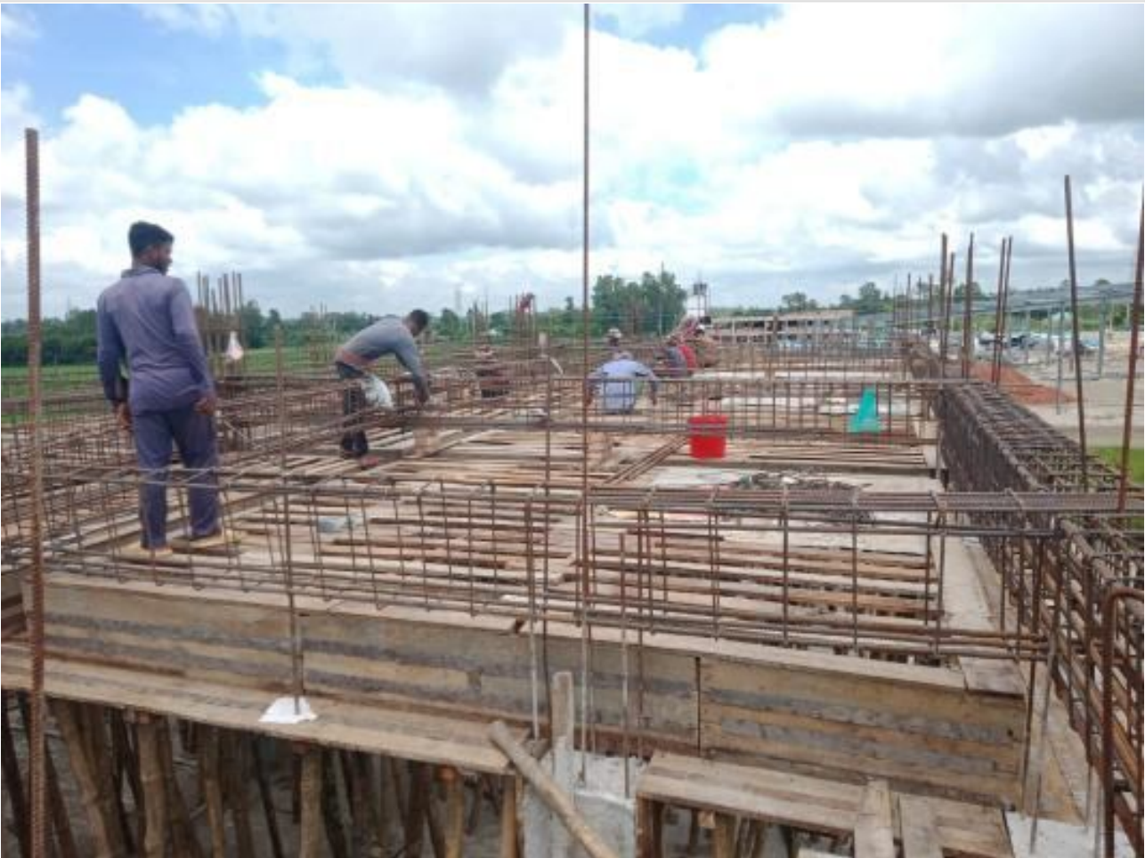
Dorm. Bldg. 2nd floor Rebar work on 07-09-23
