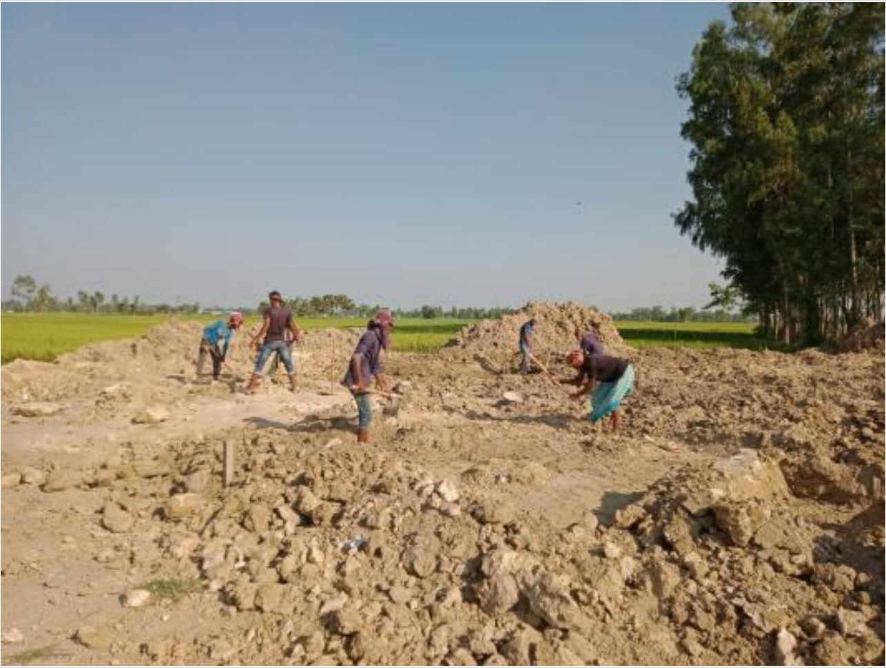
Earth cutting for dorm. Bldg. on 06-05-23
