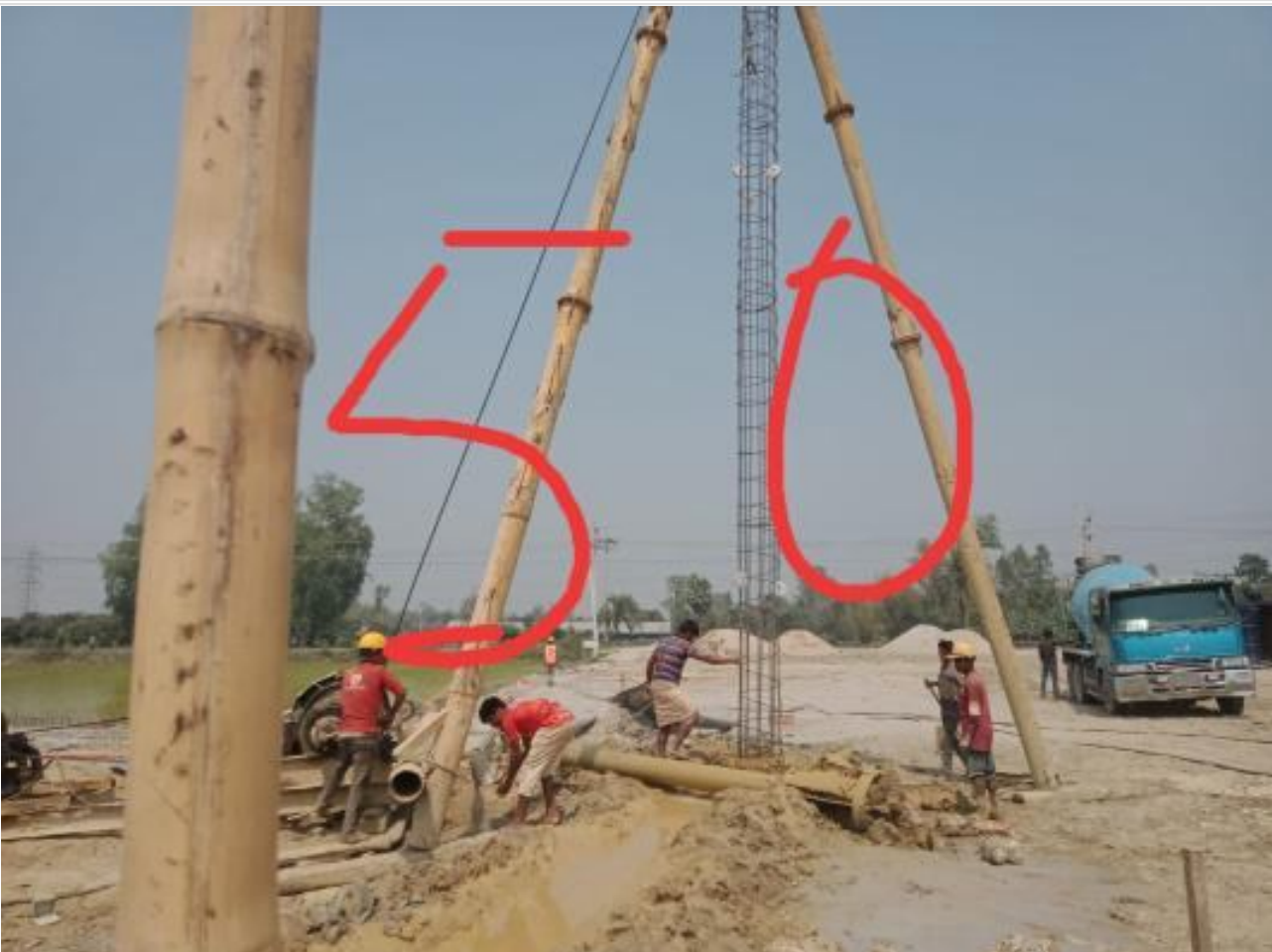
Ready mix concreting of pile on 08-03-23
