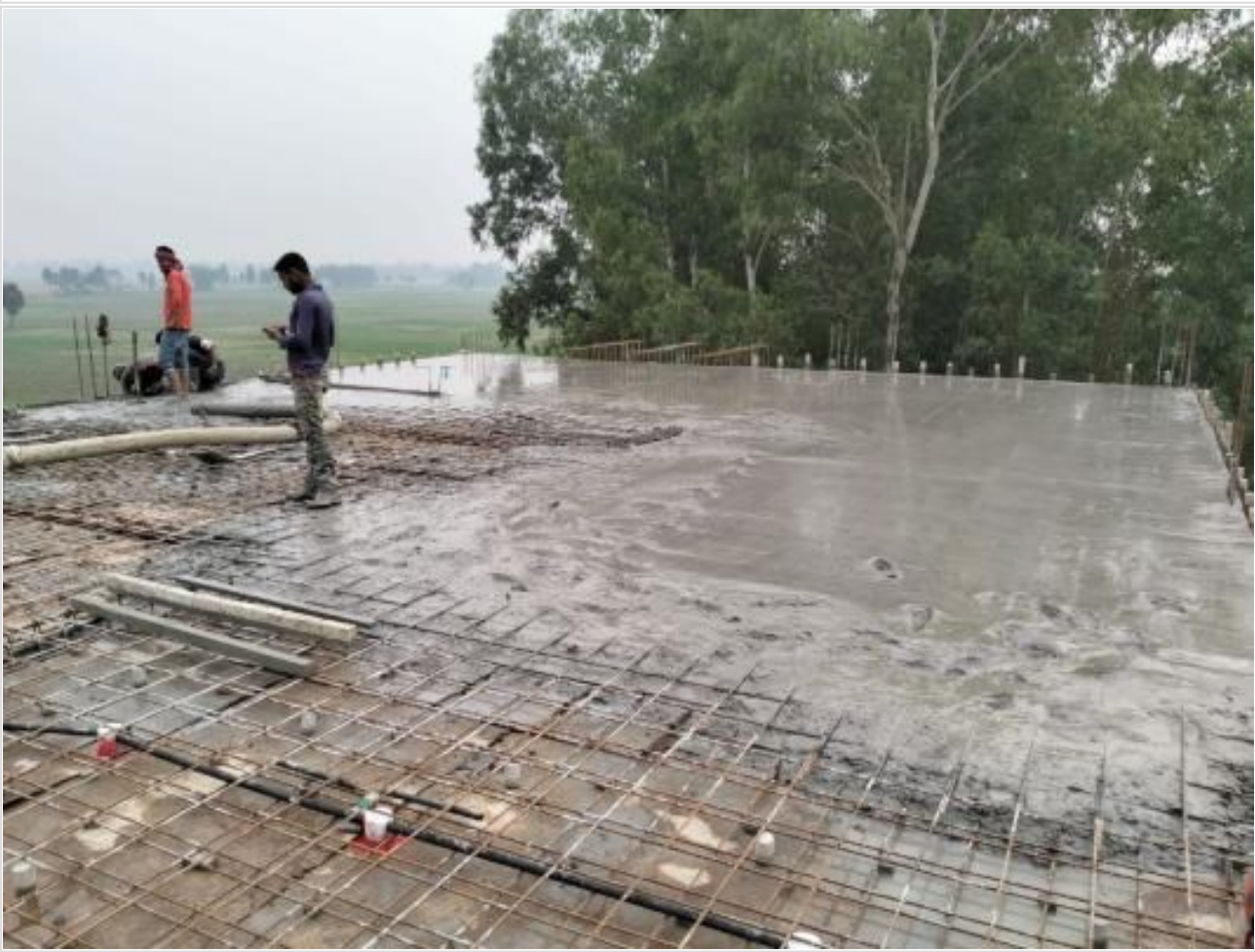
Dormitory-3rd Floor Slab Concreting on 23-12-23
