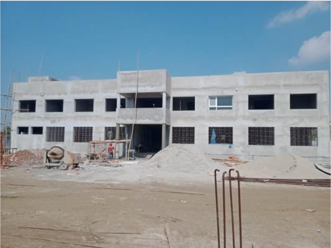
Comp. Bldg. on 26-10-23
