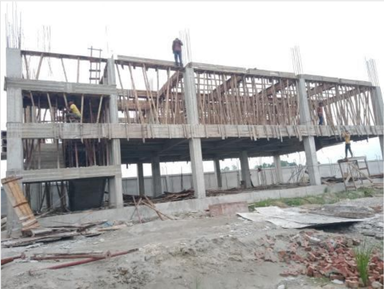
Dorm. Bldg. 2nd floor Shuttering work on 04-09-23
