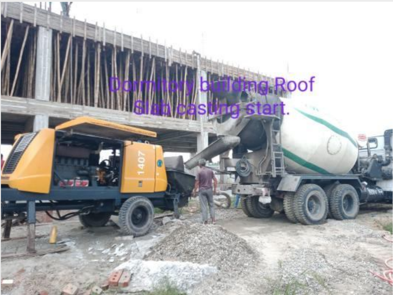
Dorm. Bldg. 2nd floor concreting work on 16-09-23
