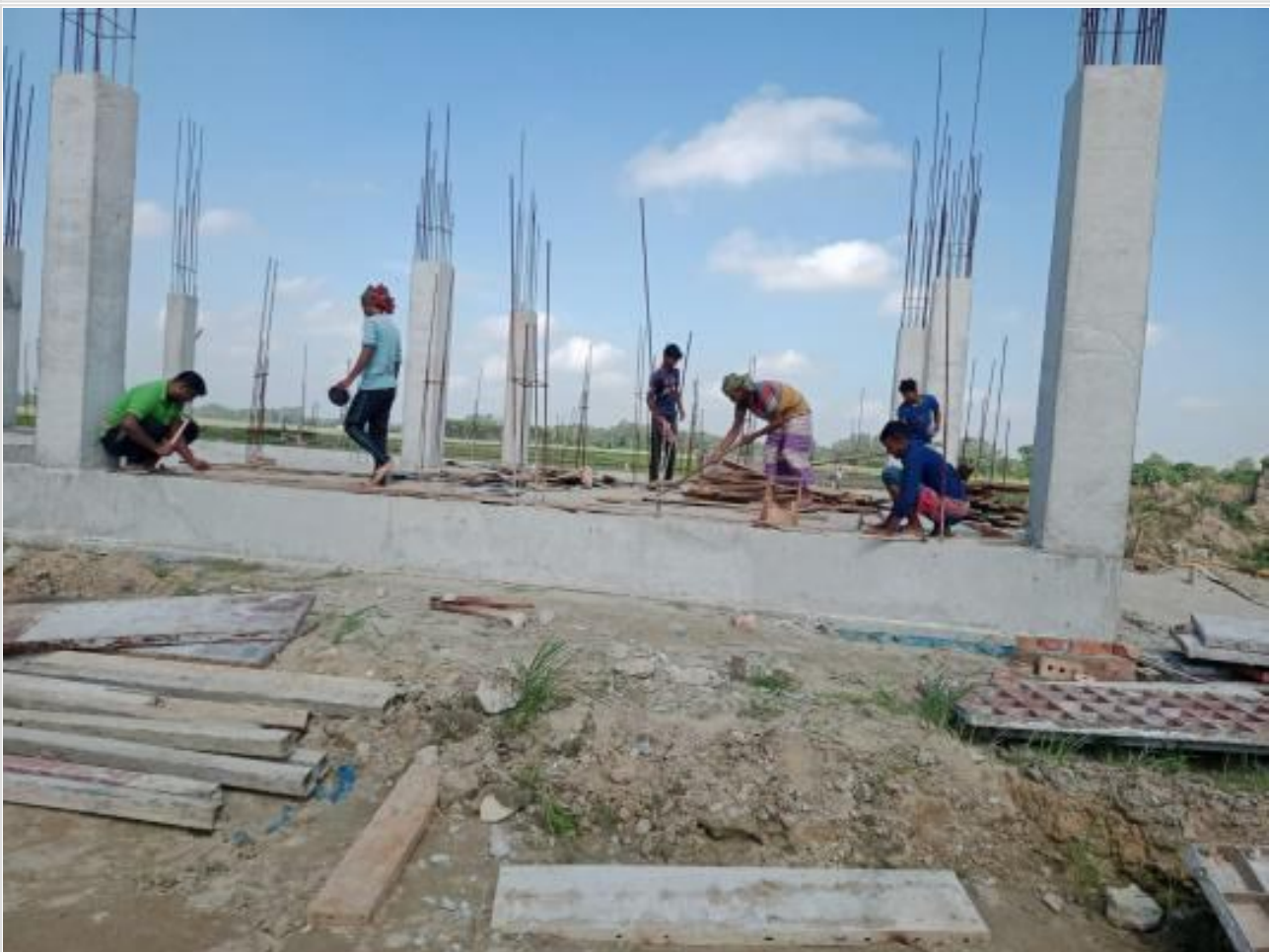
Dorm. Bldg. Floor levelling work on 20-07-23
