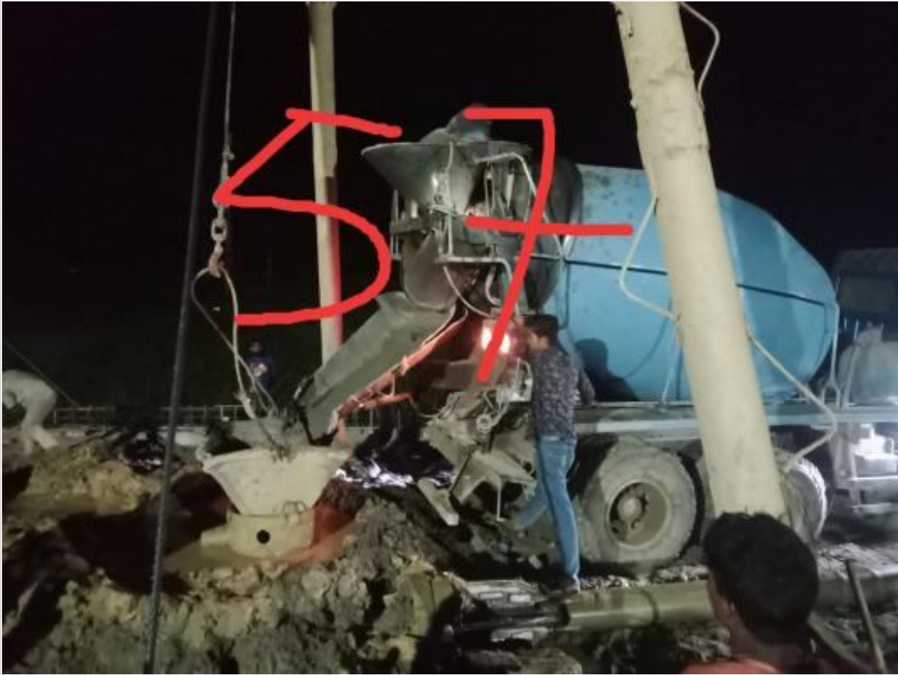
Ready mix concreting of pile on 12-03-23
