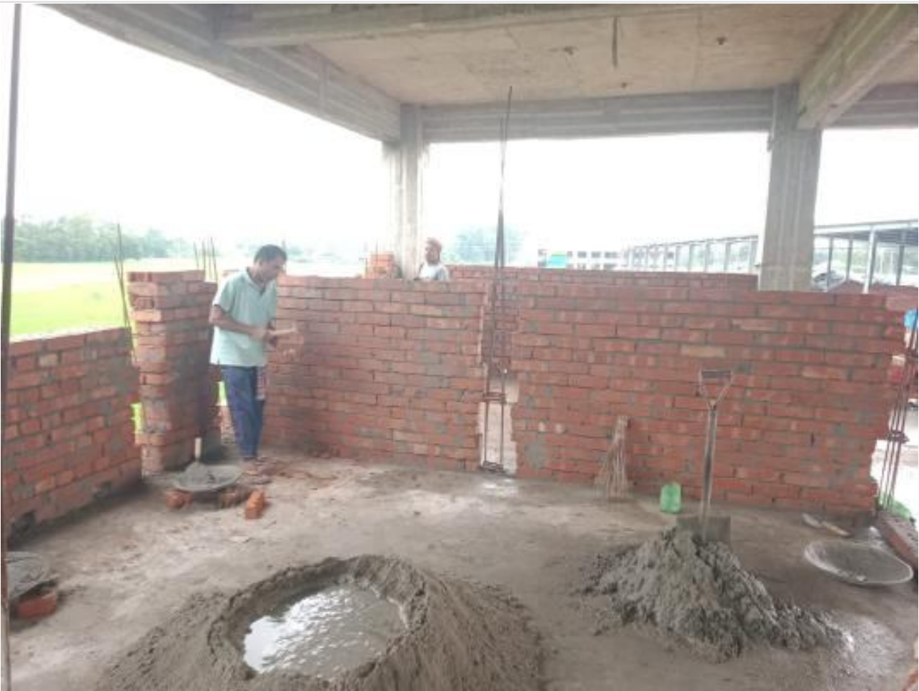
Dorm. 1st floor brick work on 04-10-23
