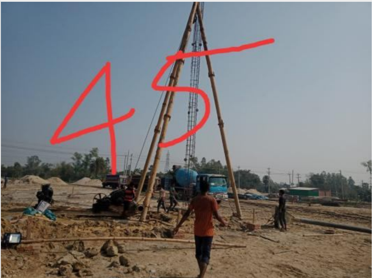
Com. Bldg. 45 Pile Boring on 06-03-23
