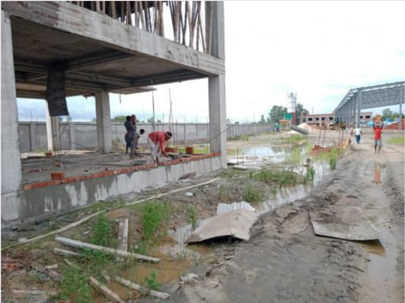
Dormitory GF-Brick Work on 20-09-23
