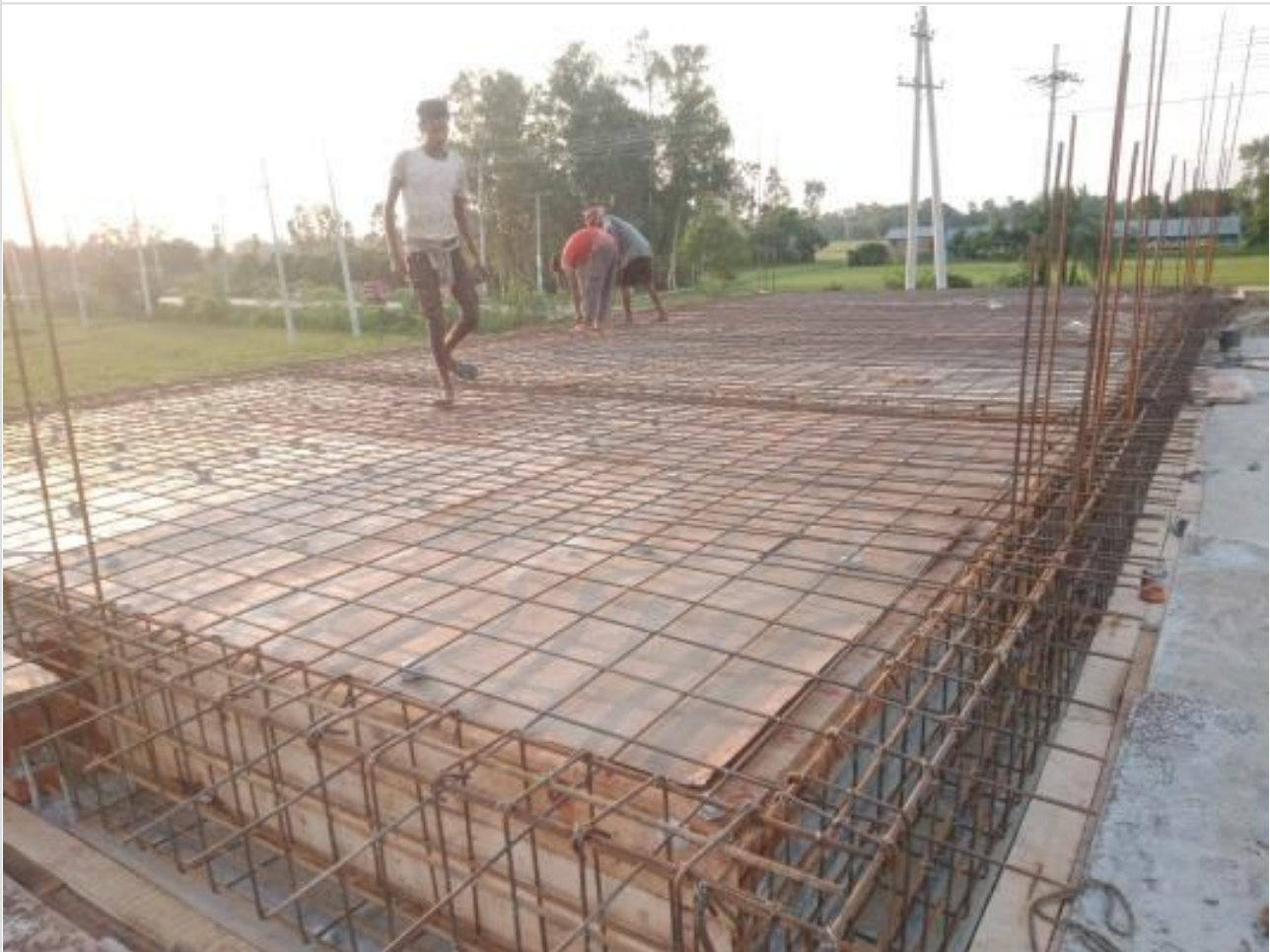
Gate House work on 25-06-23
