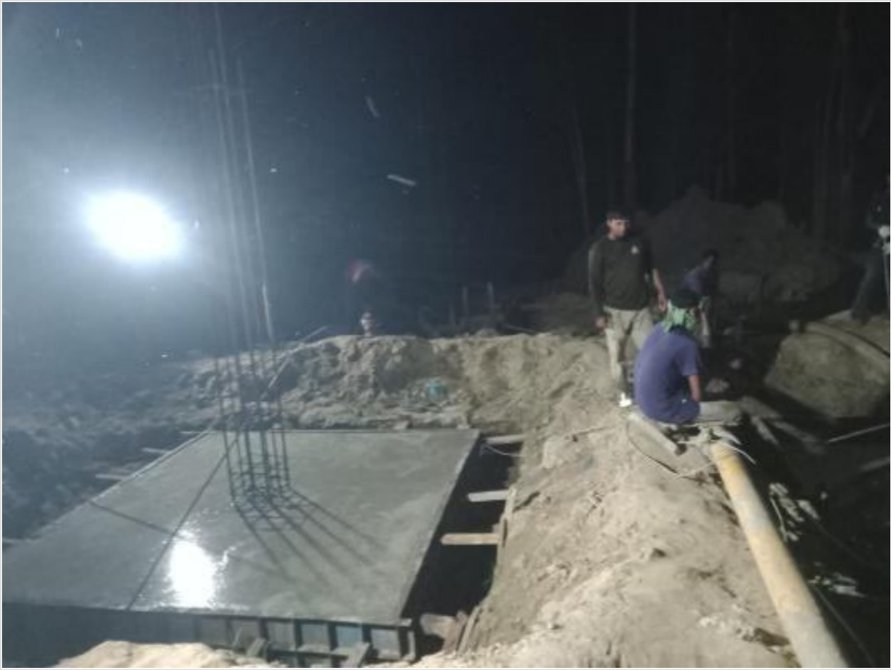
Pile Cap concreting. on 29-05-23
