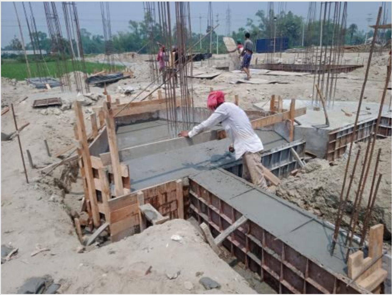
Pile cap concreting on 18-04-23
