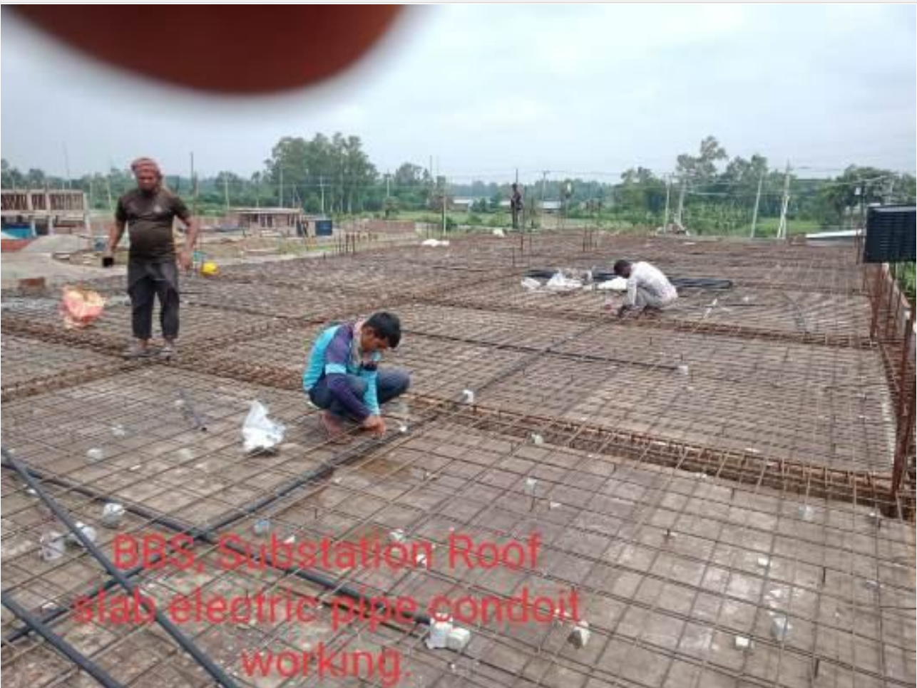
Sub-station-Electrical Pipe Work on 22-07-23
