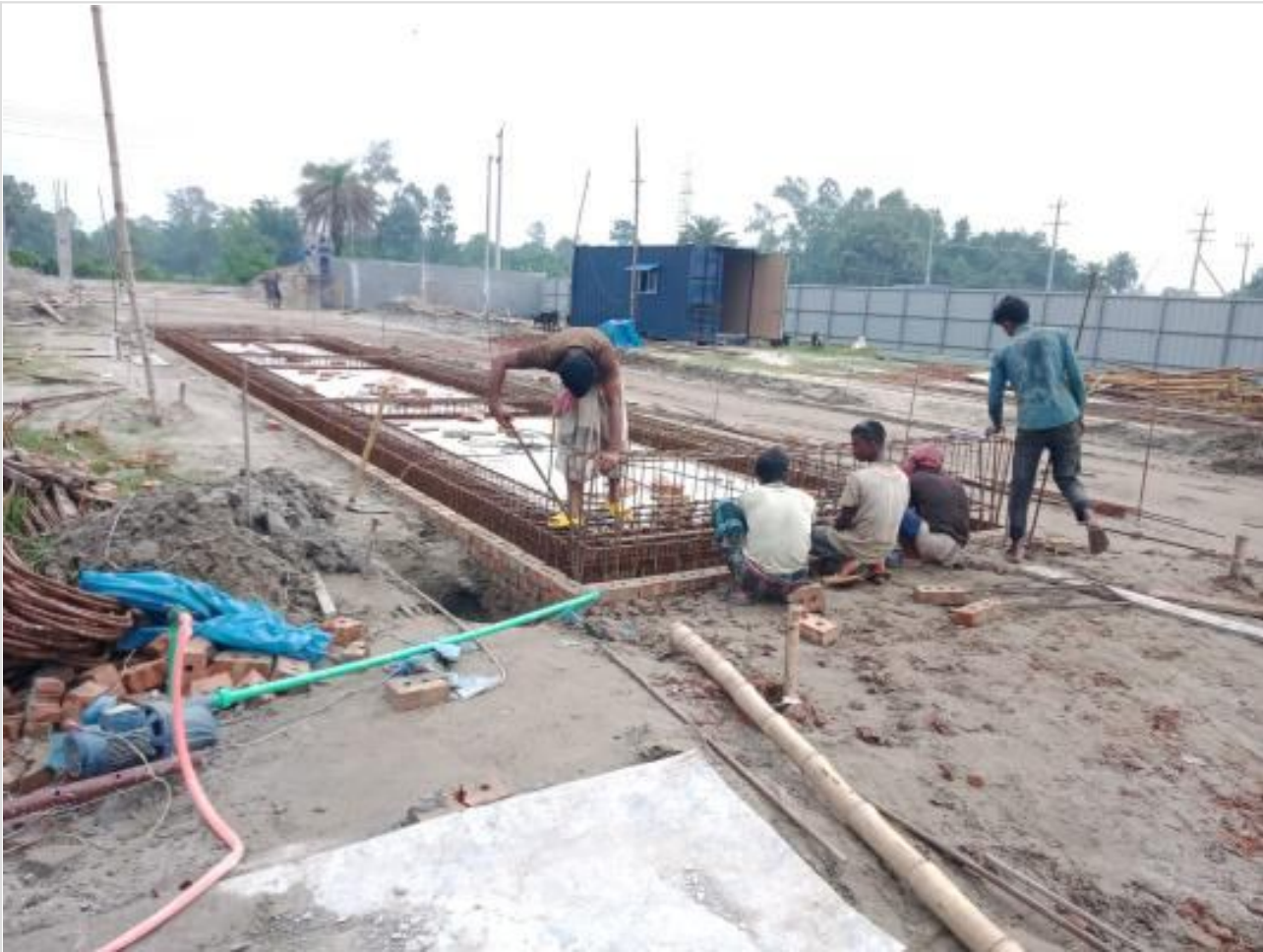
Weighing bridge re-bar work on 11-08-23
