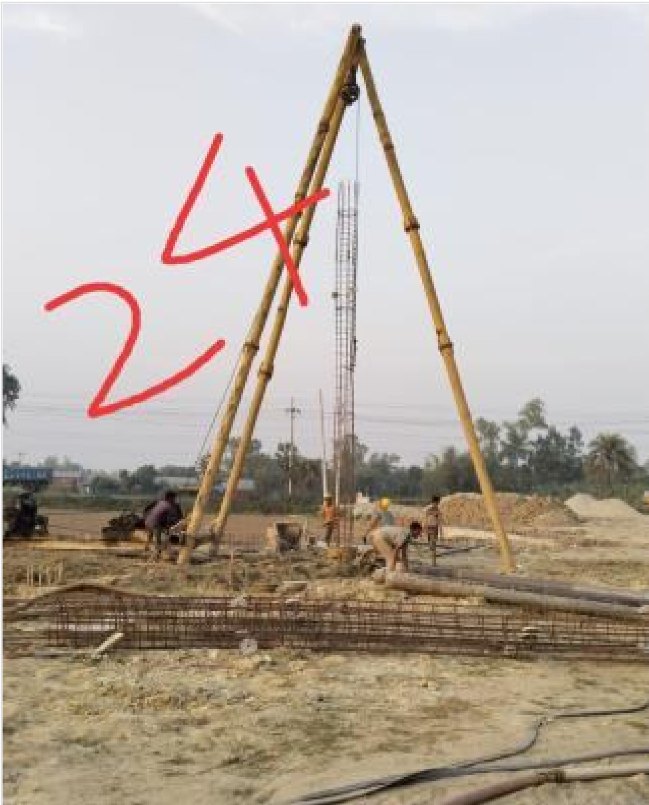
Com. Bldg. 24th pile boring on 24-02-23
