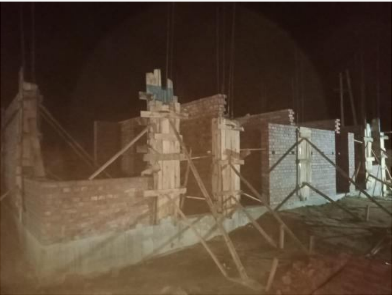
Gate House column casting on 18-06-23
