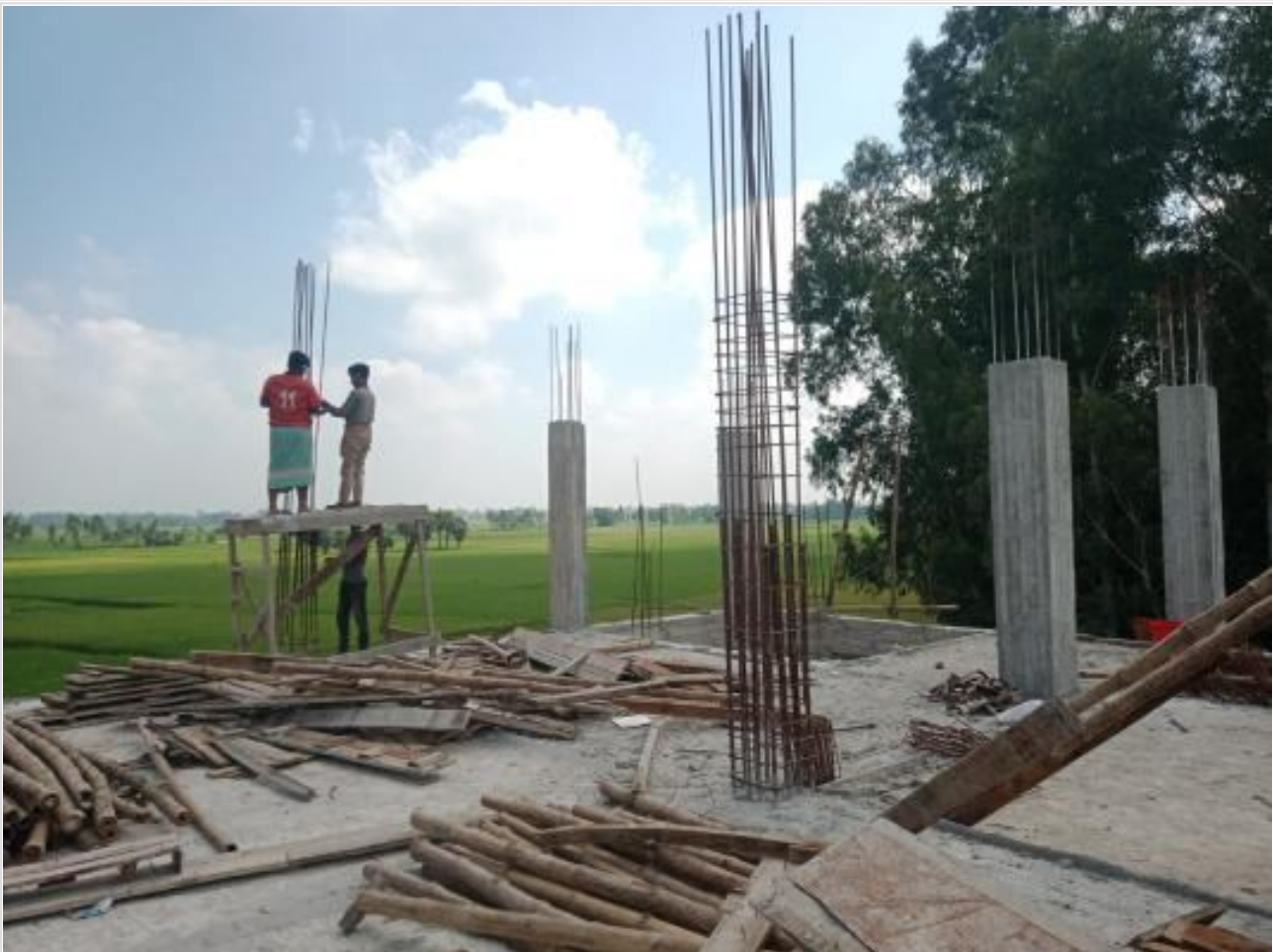
Dorm. Bldg. 2nd floor column work on 25-10-23
