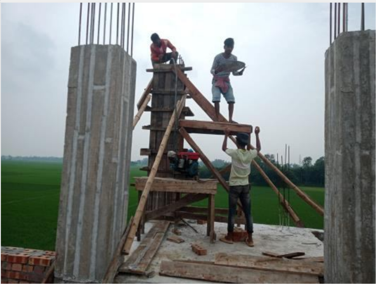
Comp. Bldg Column casting on 27-08-23
