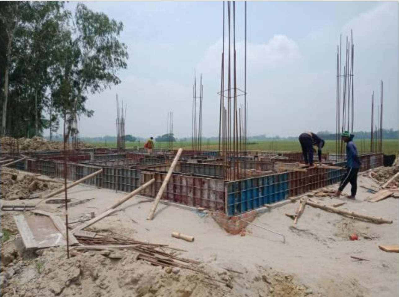
Dorm. Bldg. GB shuttering on 09-06-23
