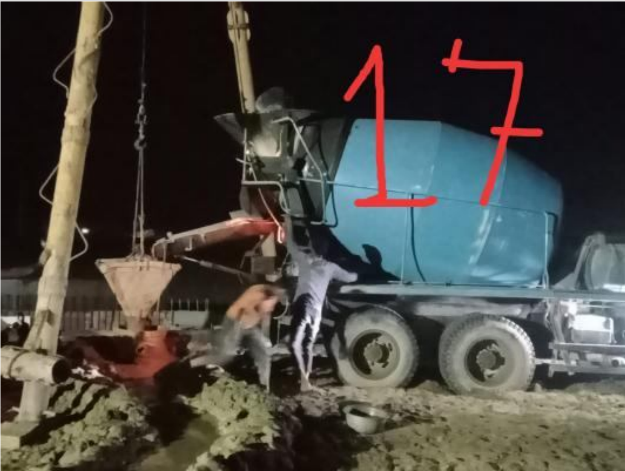
Ready mix concreting of pile on 21-02-23
