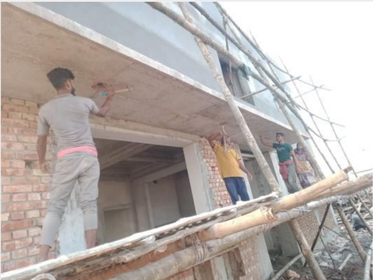
Comp. Bldg. Outside plaster work on 13-10-23
