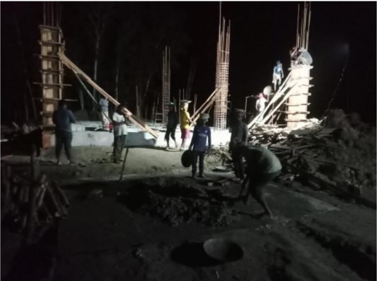
Dorm. Bldg. Column casting on 18-06-23
