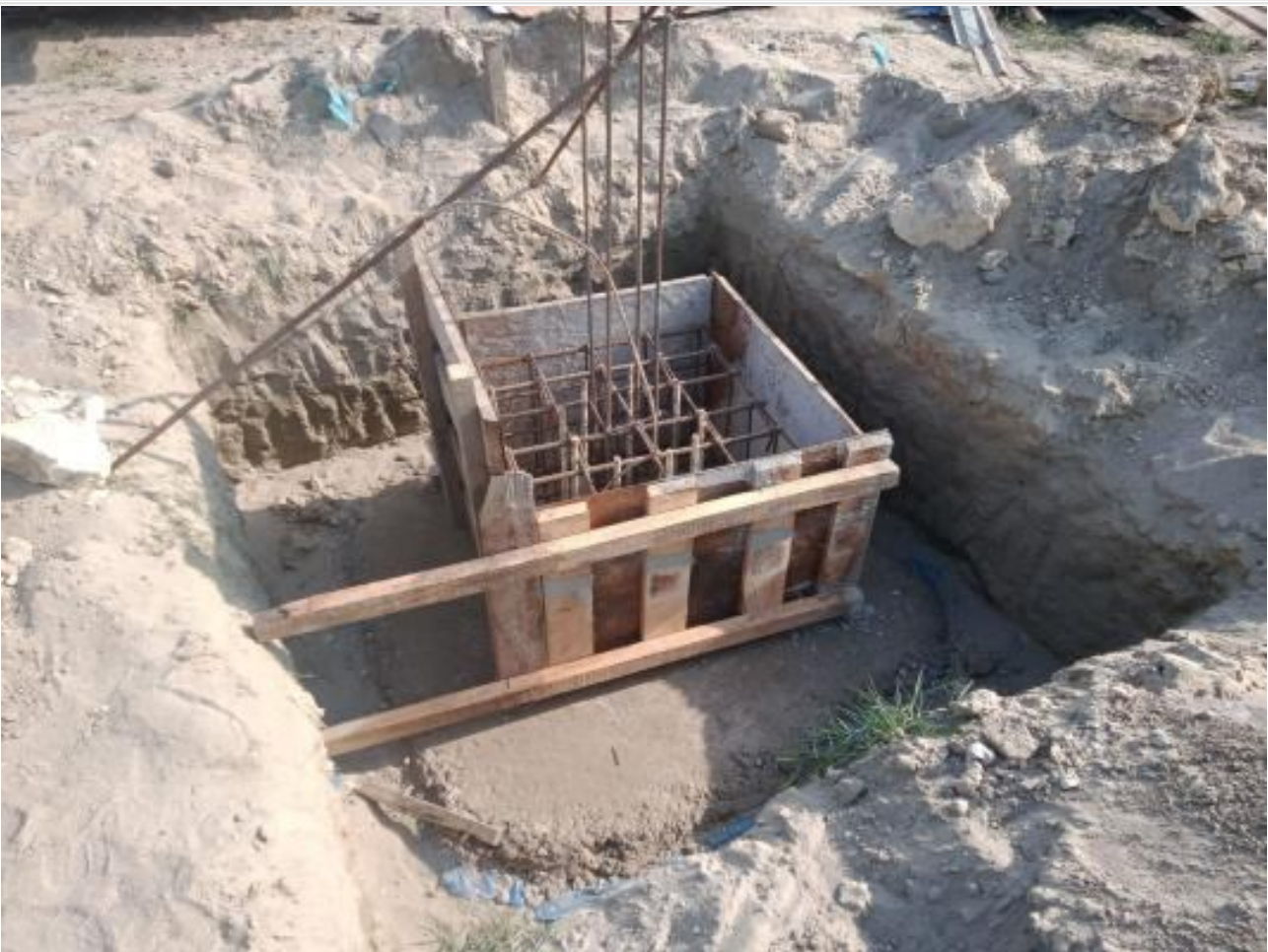
G. House Pile cap work on 09-05-23
