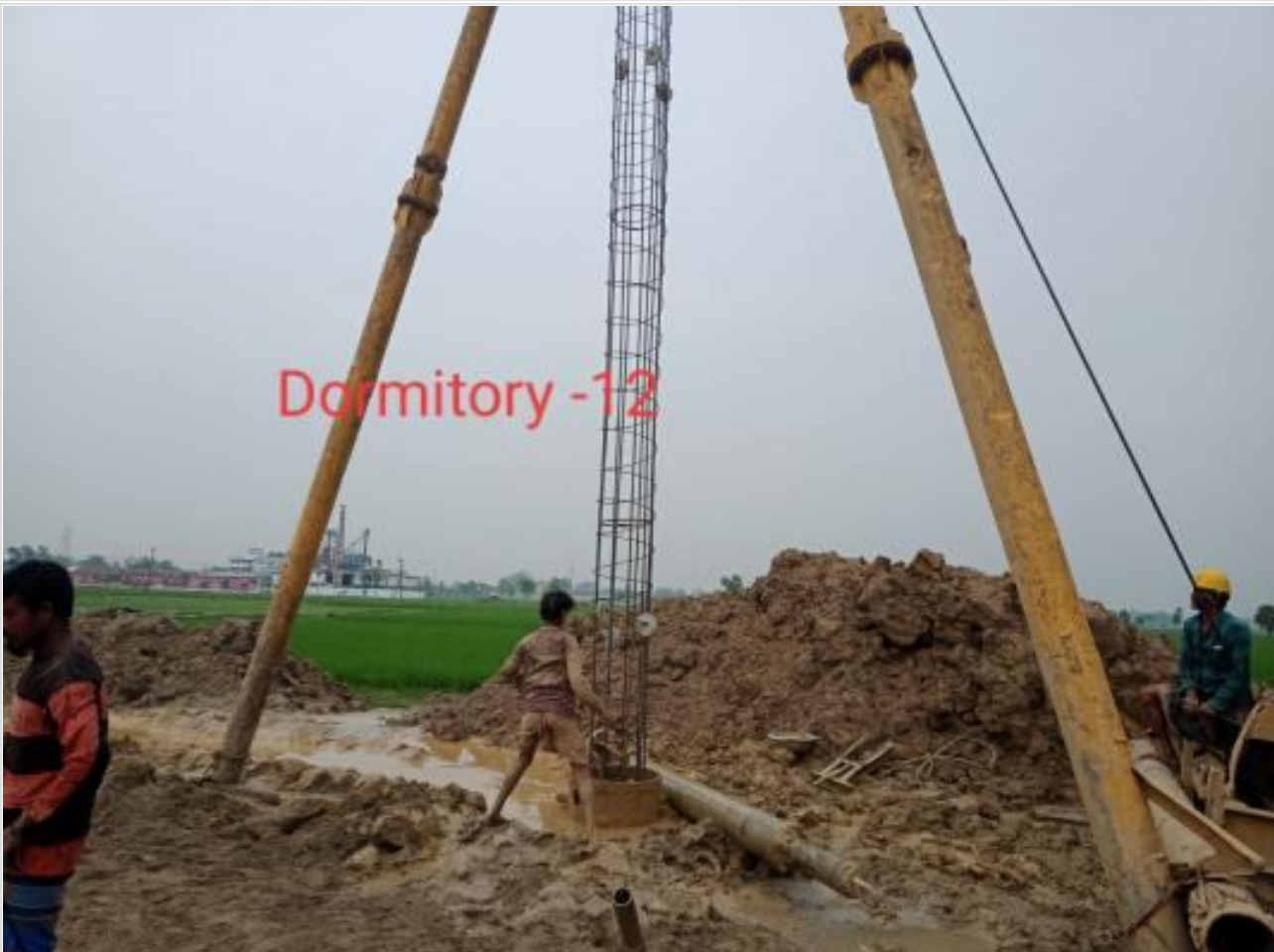
Dorm. Bldg. 10th pile concreting on 30-03-23
