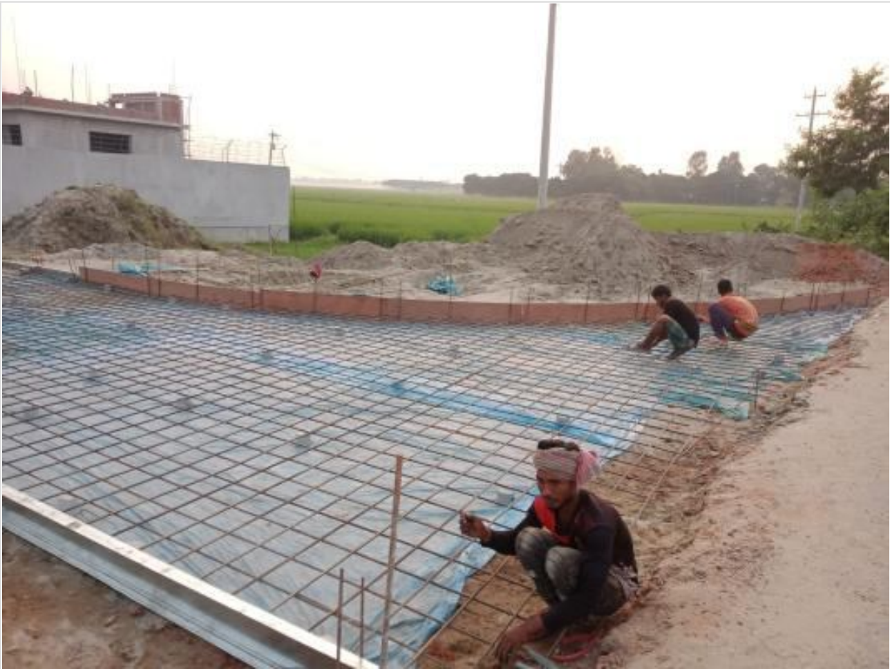
Road work on 15-10-23
