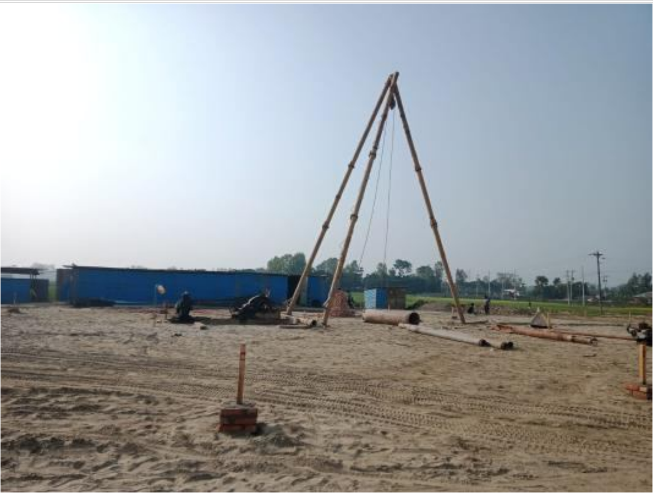
Pile Rig setting on 03-02-23
