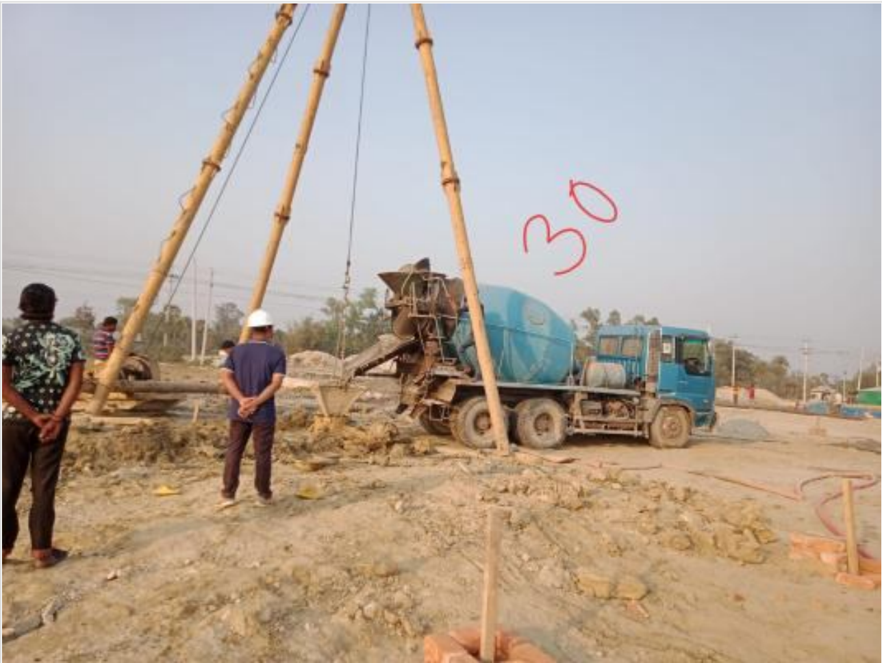
Ready mix concreting of pile on 26-02-23
