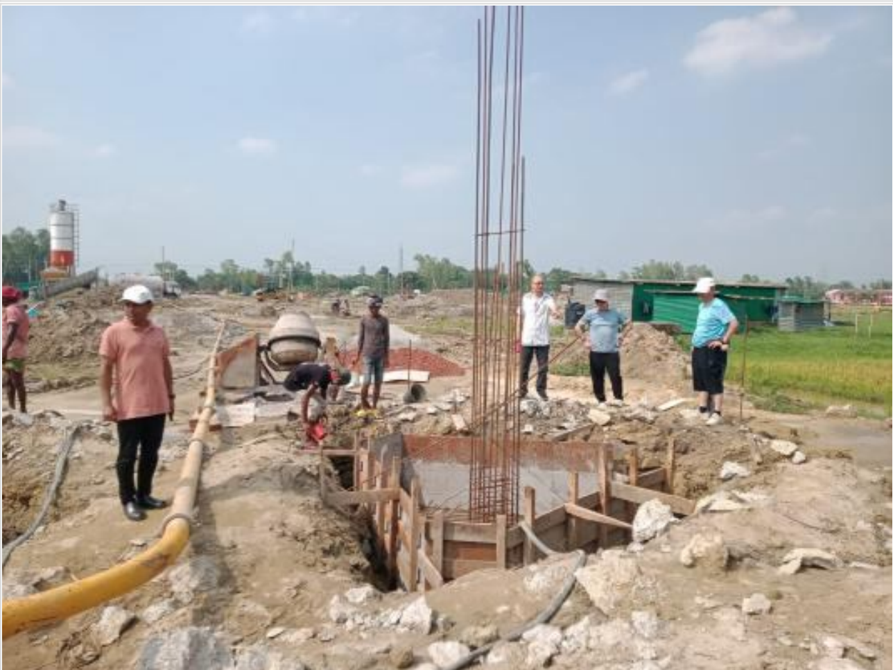
Dorm. Bldg pile cap work on 26-05-23
