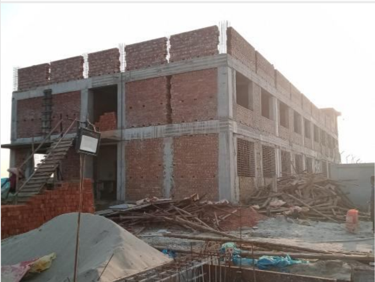
Comp. Bldg work on 15-09-23
