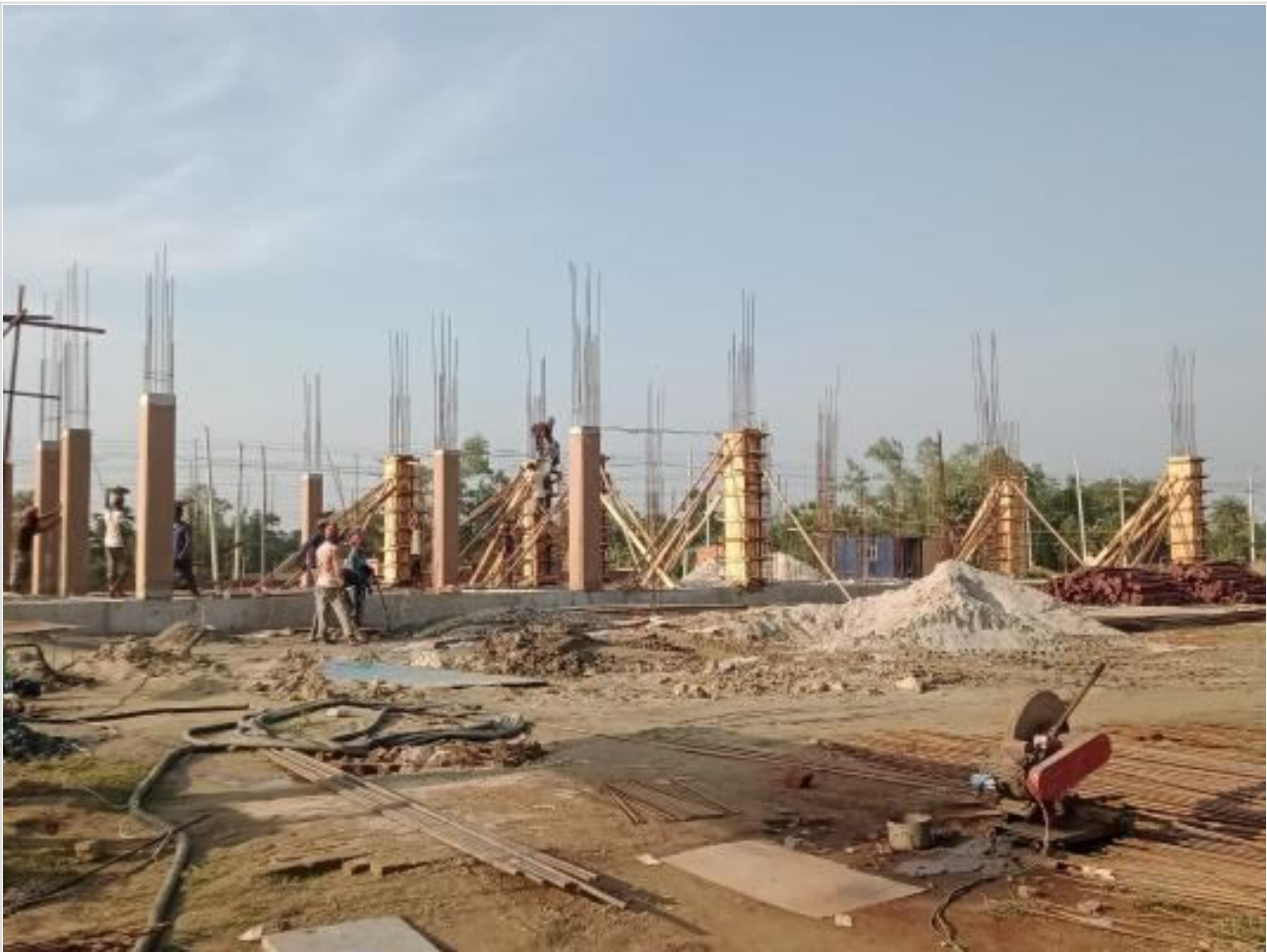
Comp. Bldg. Column shutter on 31-05-23
