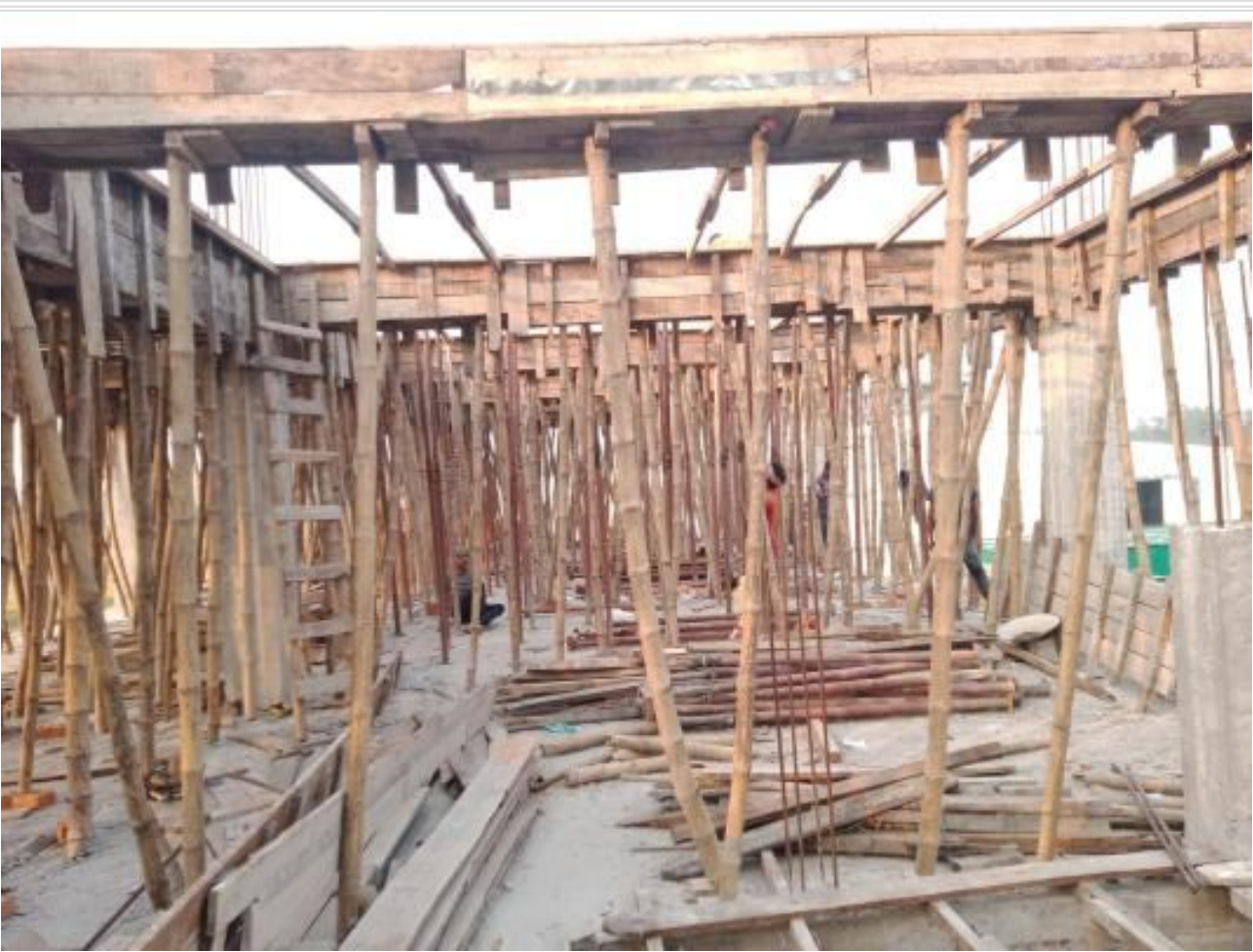
Dorm. Bldg. 3rd floor slab shuttering on 08-11-23
