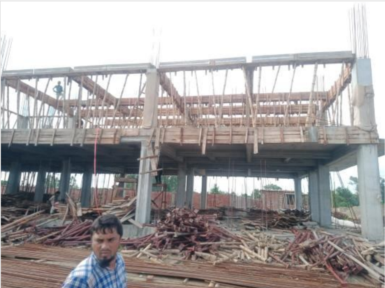
Comp. Bldg. Slab beam shuttering on 17-07-23
