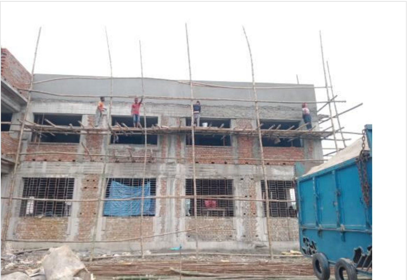
Comp. Bldg. Outside plaster work on 10-10-23
