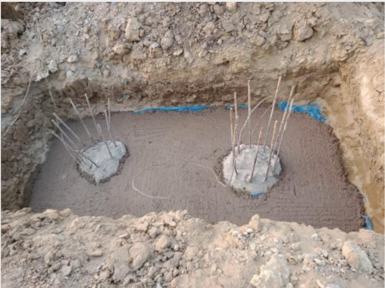
Pile cap bottom cc work of Dorm. Bldg on 11-05-23
