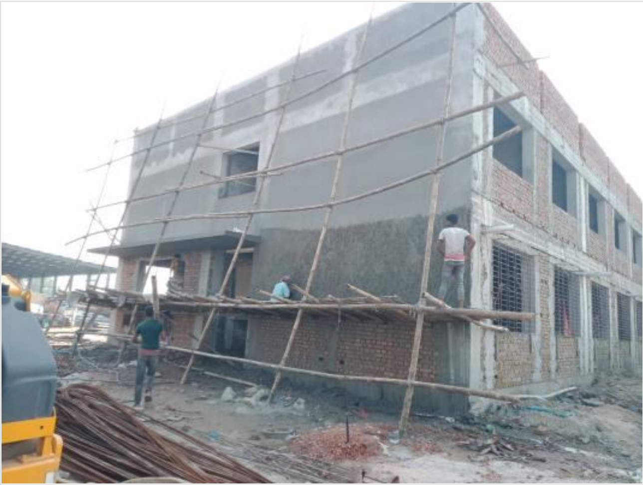
Comp. Bldg. Outside plaster work on 14-10-23
