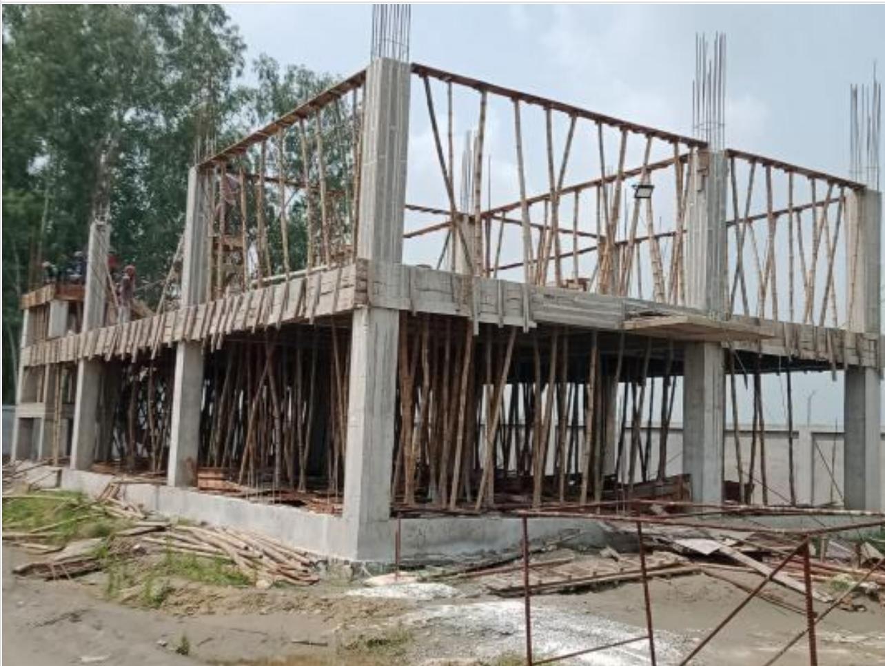
Dorm. Bldg. 2nd floor shuttering on 29-08-23
