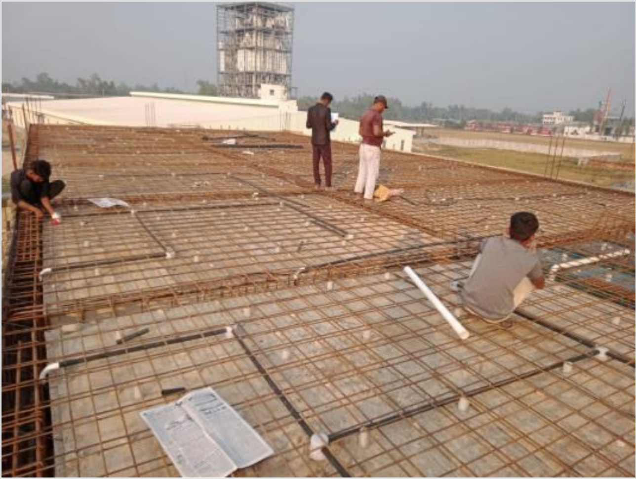
Dormitory-3rd Floor Slab Re-bar Work on 18-12-23
