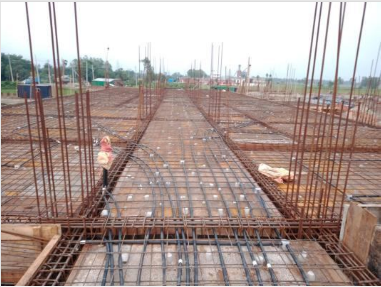
Comp. Bldg. Slab Ready for Concrete on 22-06-23
