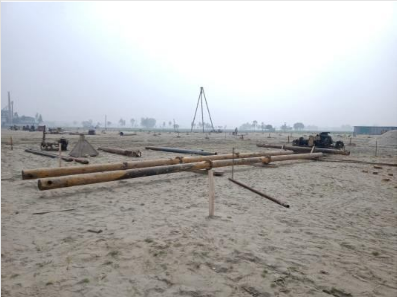
Pile Rig Installing on 31-01-23
