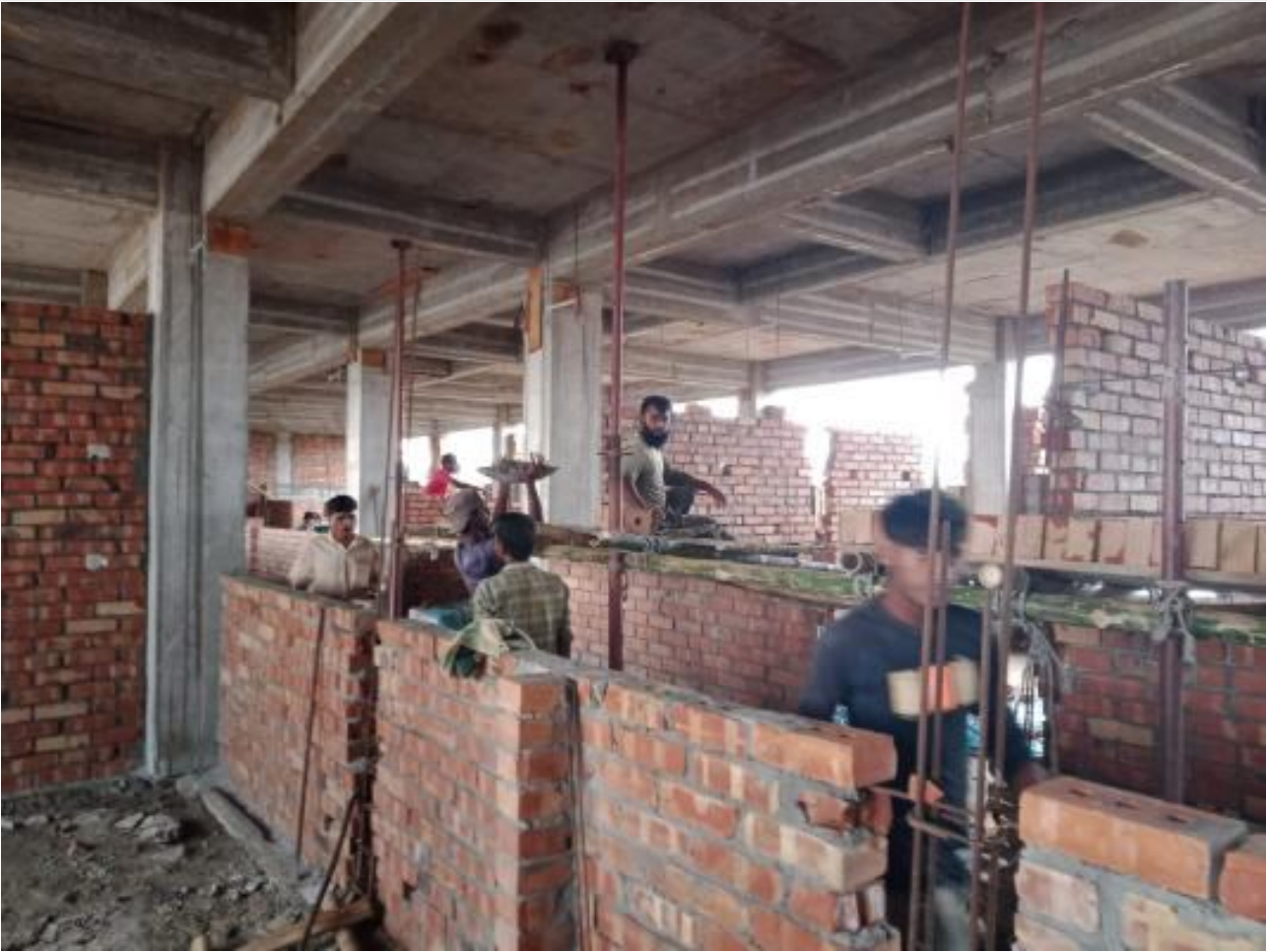
Tie column work at brick wall on 02-08-23
