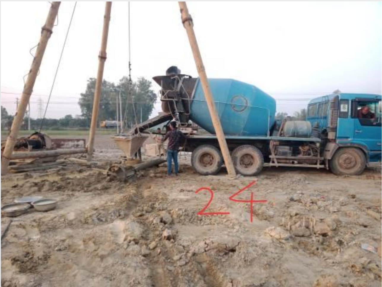
Ready mix concreting of pile on 24-02-23
