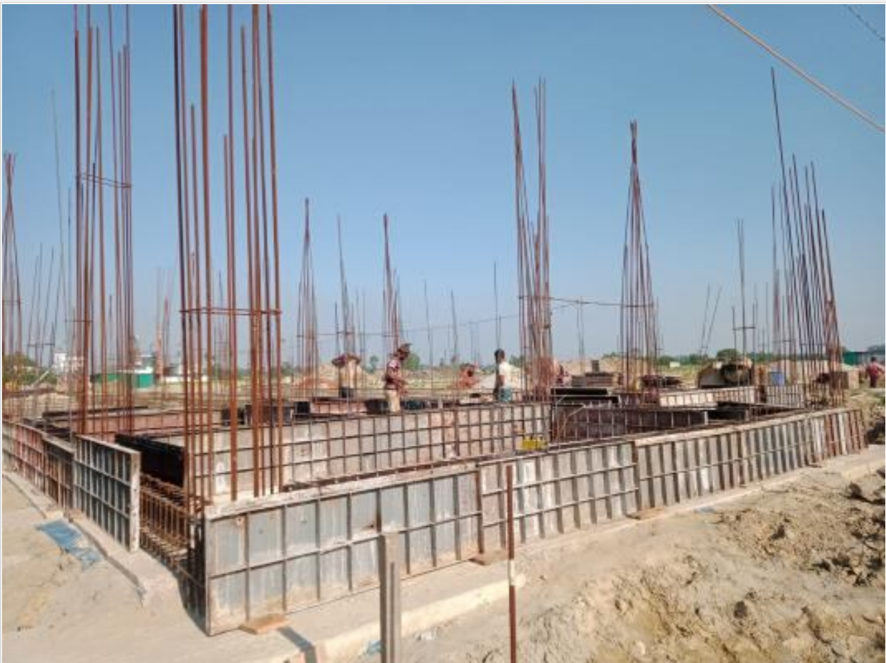
Comp. GB Shuttering on 06-05-23
