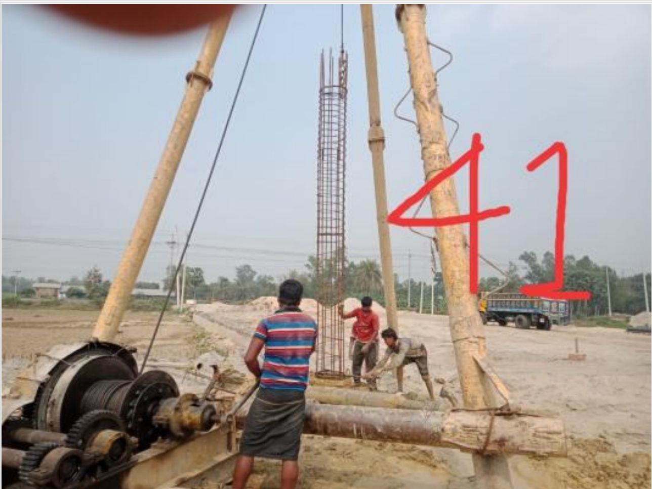
Com. Bldg. 41 Pile Boring on 03-03-23
