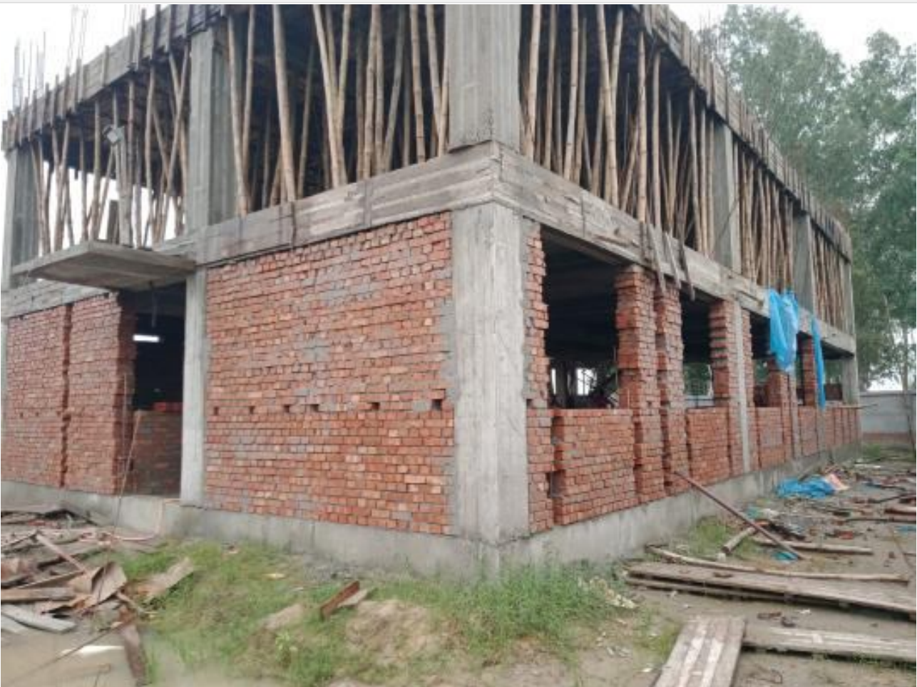
Dorm.Bldg. GF brick work on 25-09-23
