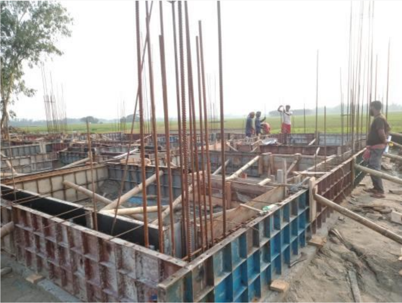
Dorm. Bldg. GB shuttering on 12-06-23
