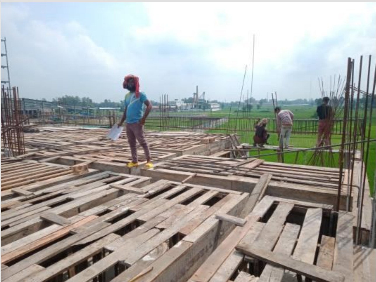
Dorm. Bldg. 2nd floor shuttering work on 06-09-23
