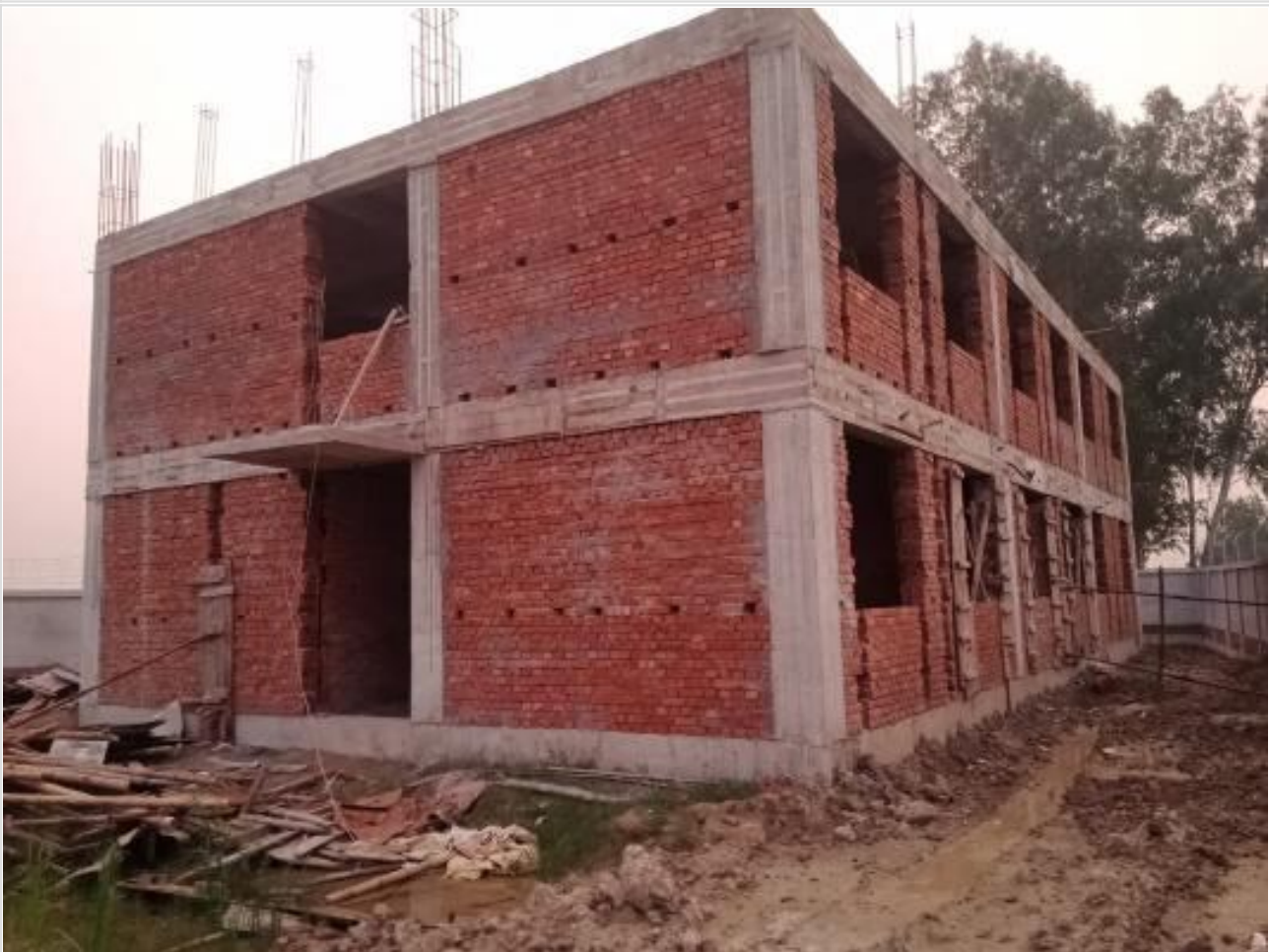
Dorm. Bldg. Brick work on 10-10-23
