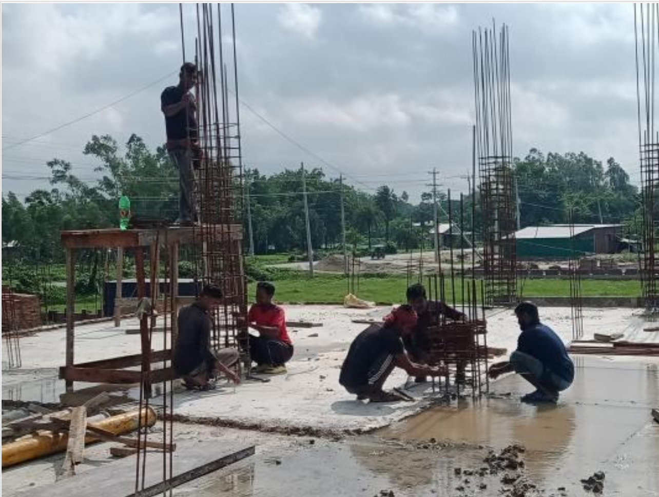
Comp. Bldg. 1st floor column work on 07-07-23
