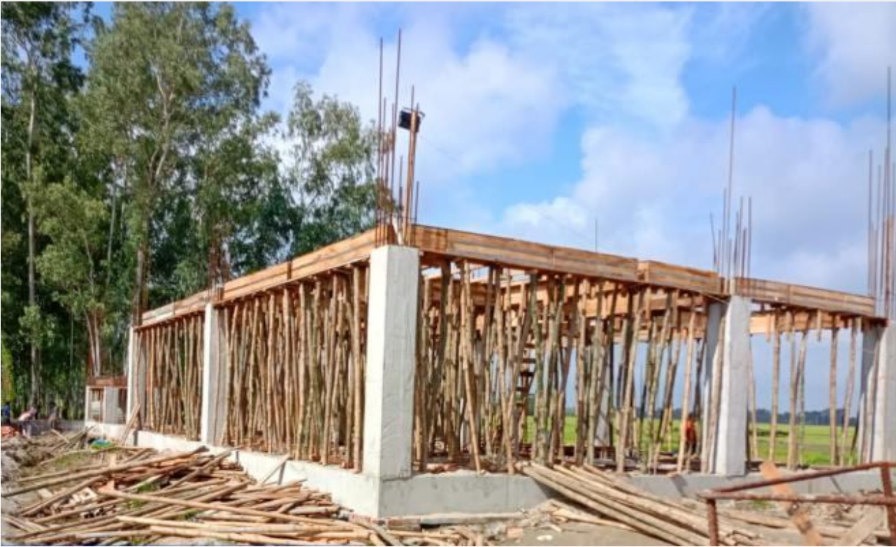
Dorm. Bldg shuttering work on 27-07-23
