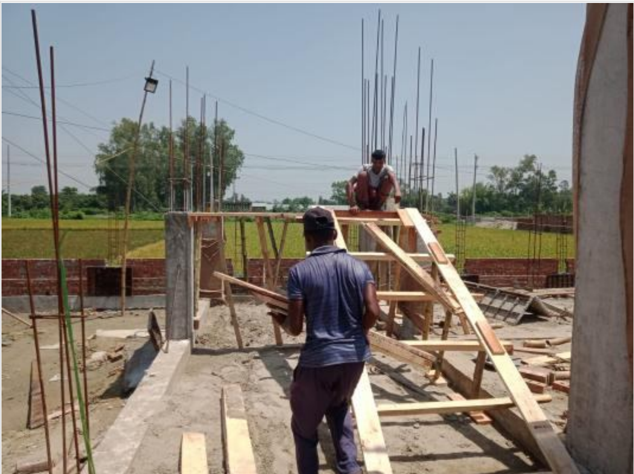
Comp. Bldg. Stair shuttering on 02-06-23
