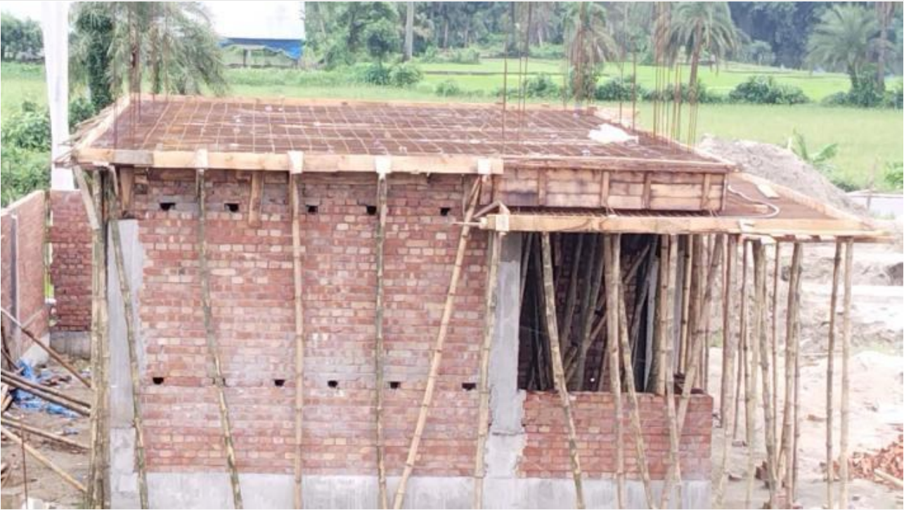
Gate House work on 04-07-23
