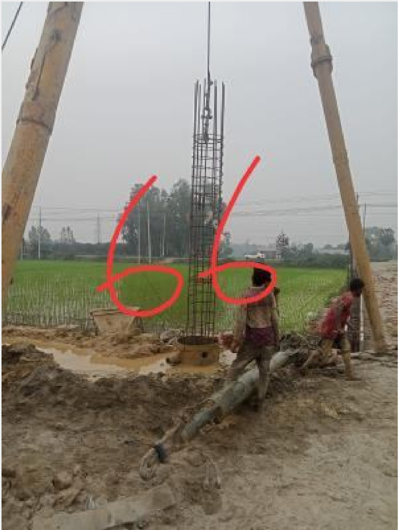
Com. Bldg. 66 Pile Boring on 16-03-23
