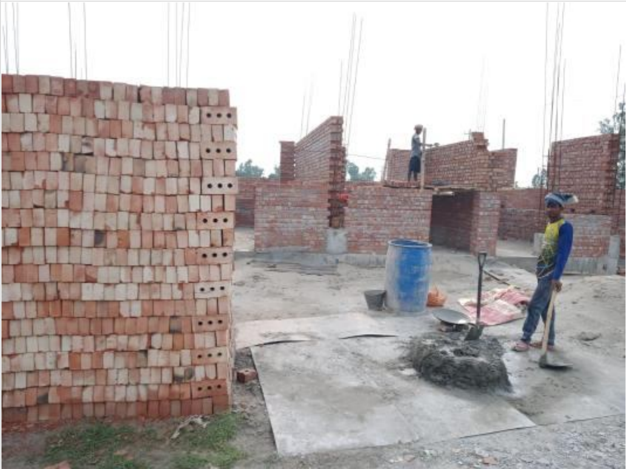
Gate house work on 15-06-23
