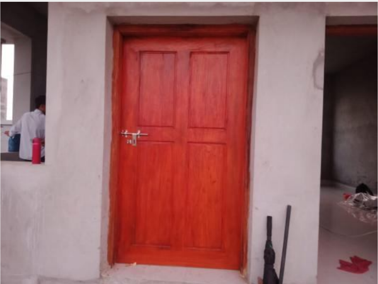
Gate House door fixed on 31-10-23
