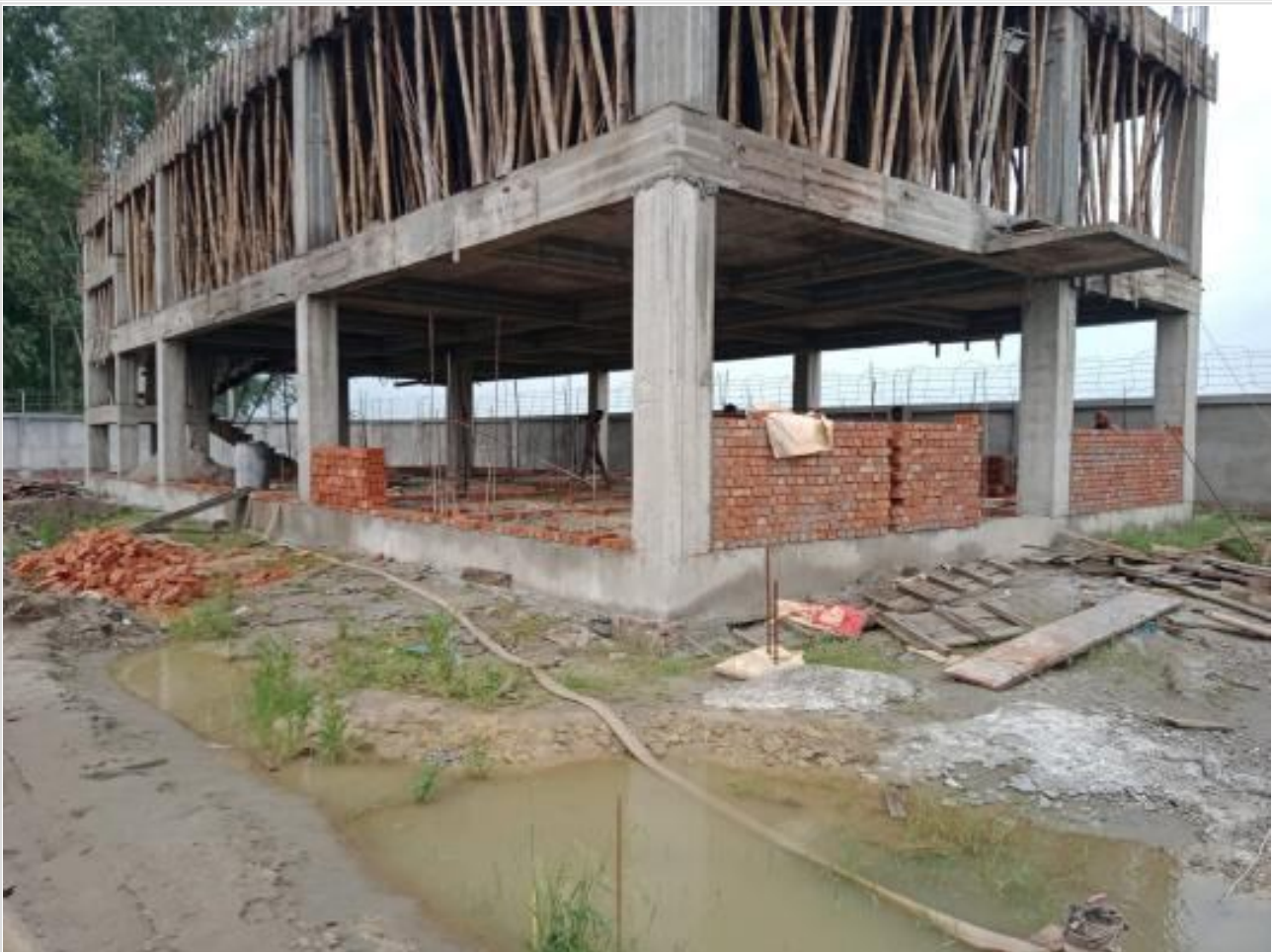
Dorm. Bldg GF Brick work on 21-09-23
