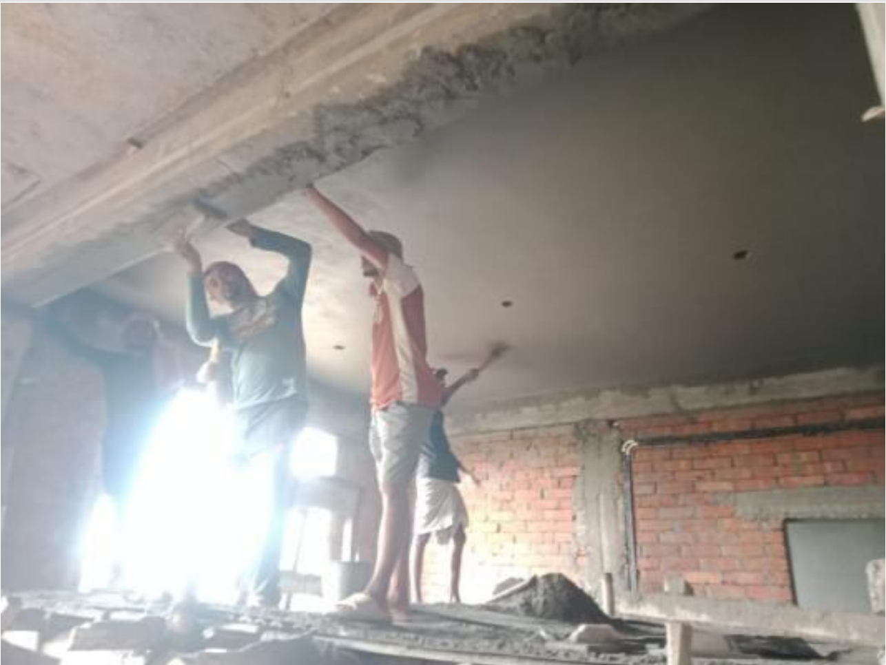
Dormitory-GF-Ceiling Plastering on 27-10-23
