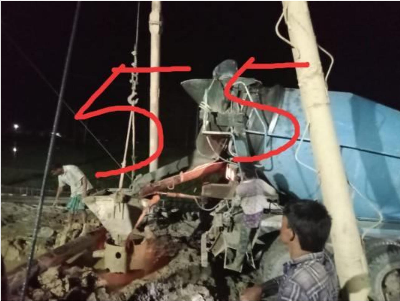
Ready mix concreting of pile on 11-03-23
