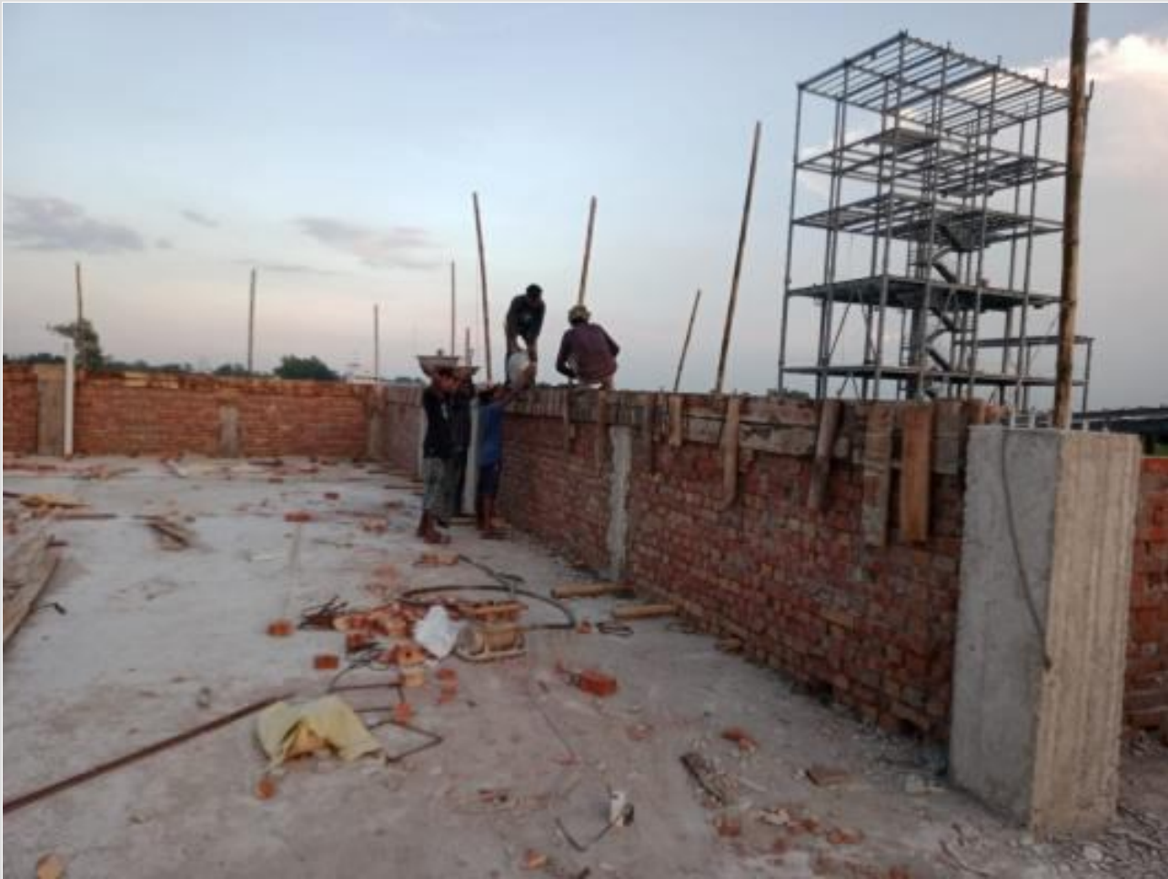
Comp. Roof top parapet work on 01-10-23
