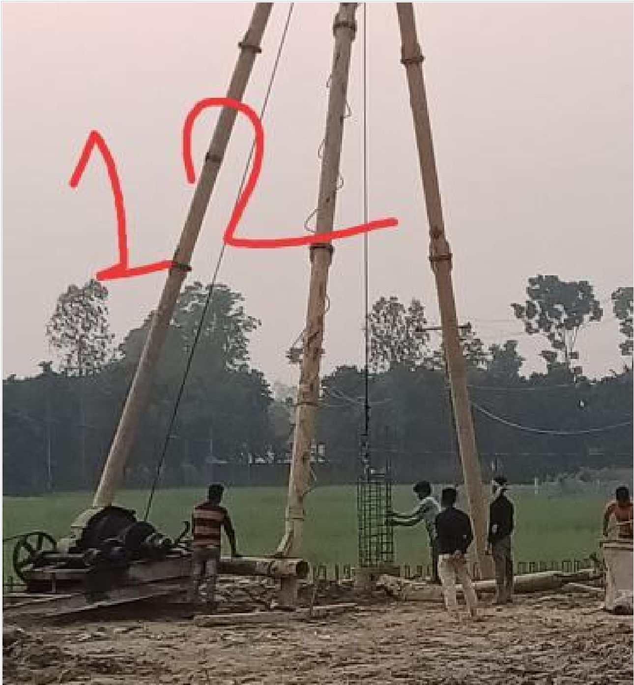
Com. Bldg. 12th pile boring on 17-02-23
