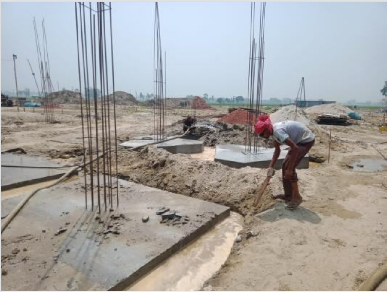
Comp. Bldg. Back filling on 19-04-23
