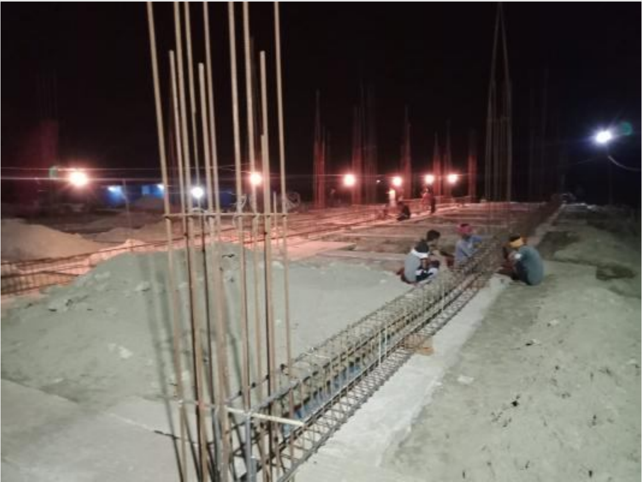
GB Re-bar work on 03-05-23
