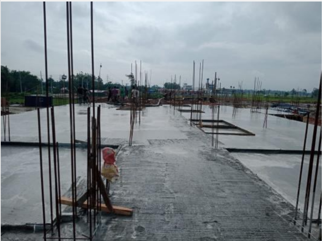
Comp. Bldg. Slab casting complete on 27-06-23
