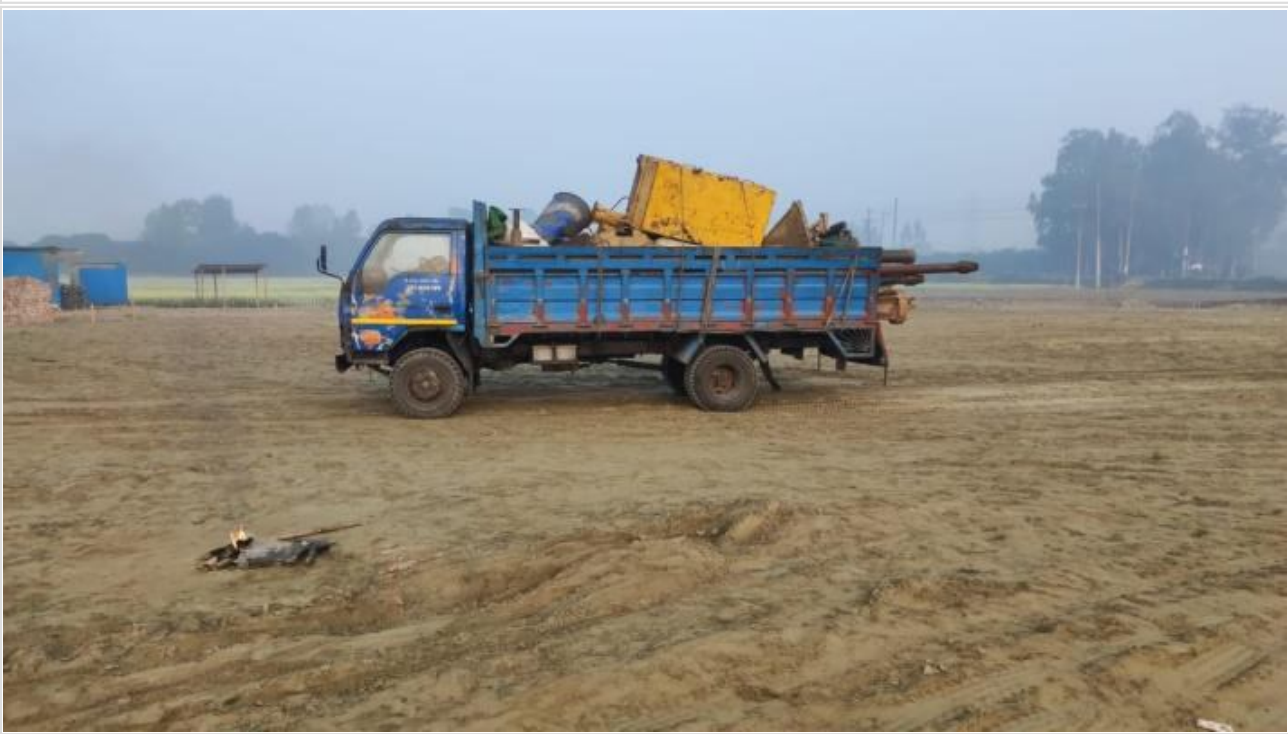
Piling Rig mobilized on 29-01-23
