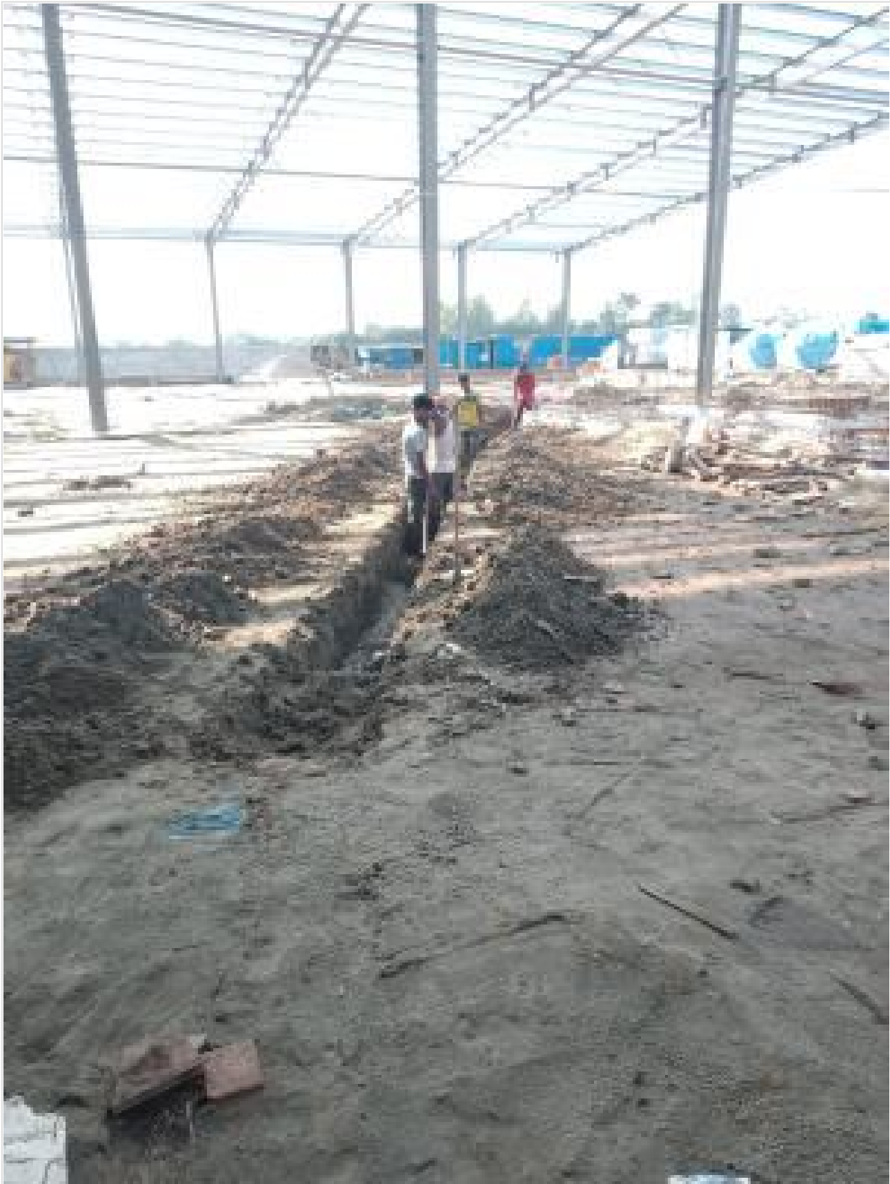
Earth cutting power cable laying on 28-09-23
