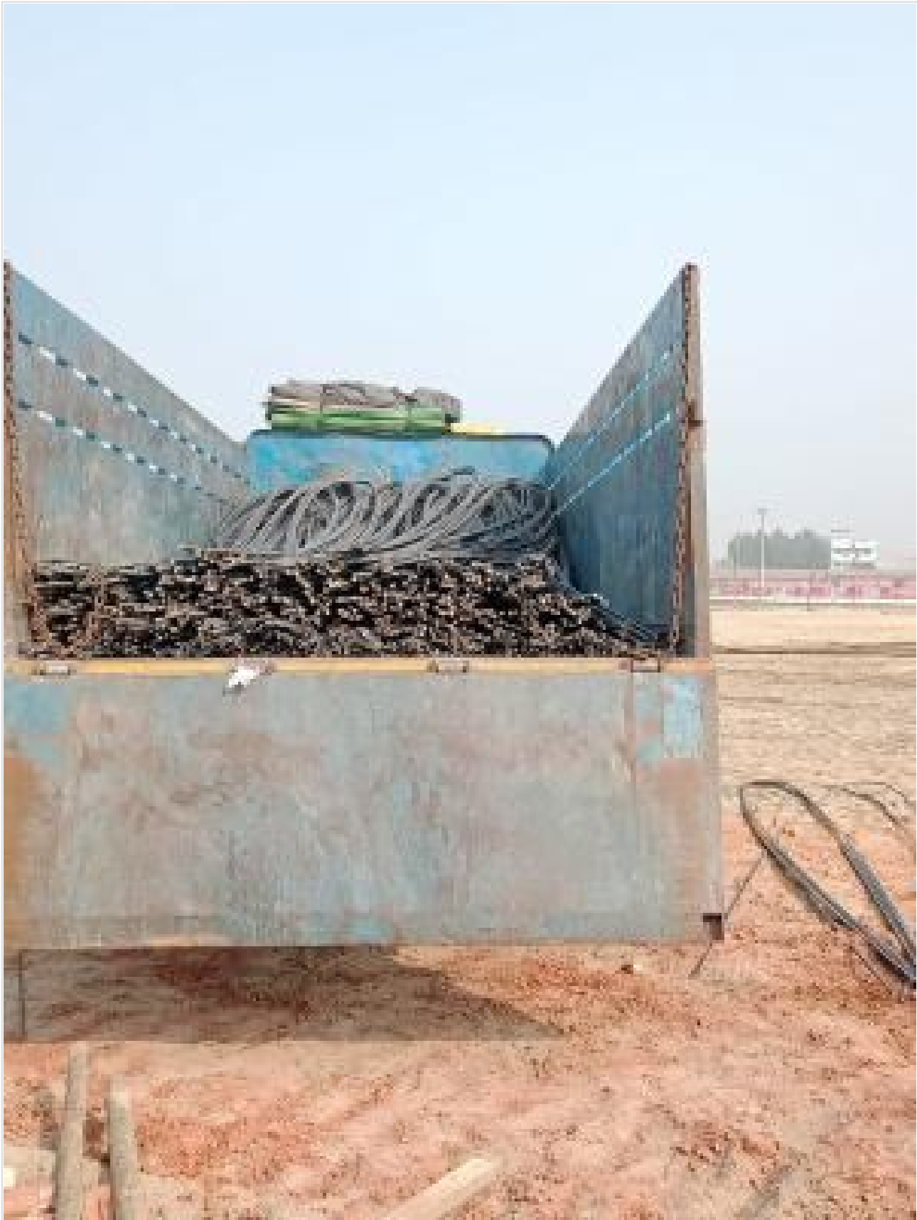
Re-bar mobilized on 21-01-23
