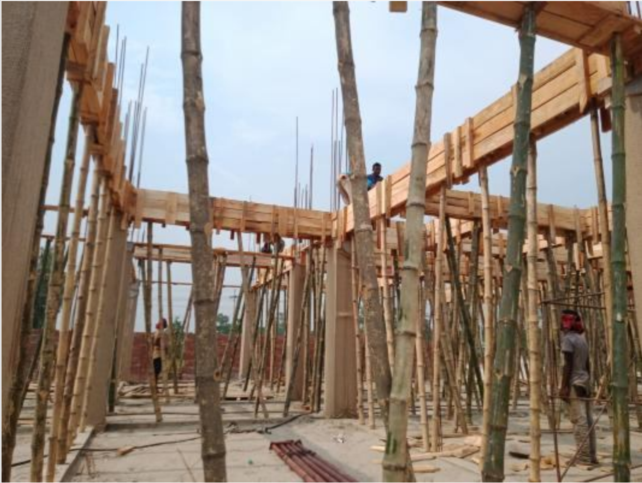
Comp. Bldg. Slab beam shuttering on 07-06-23
