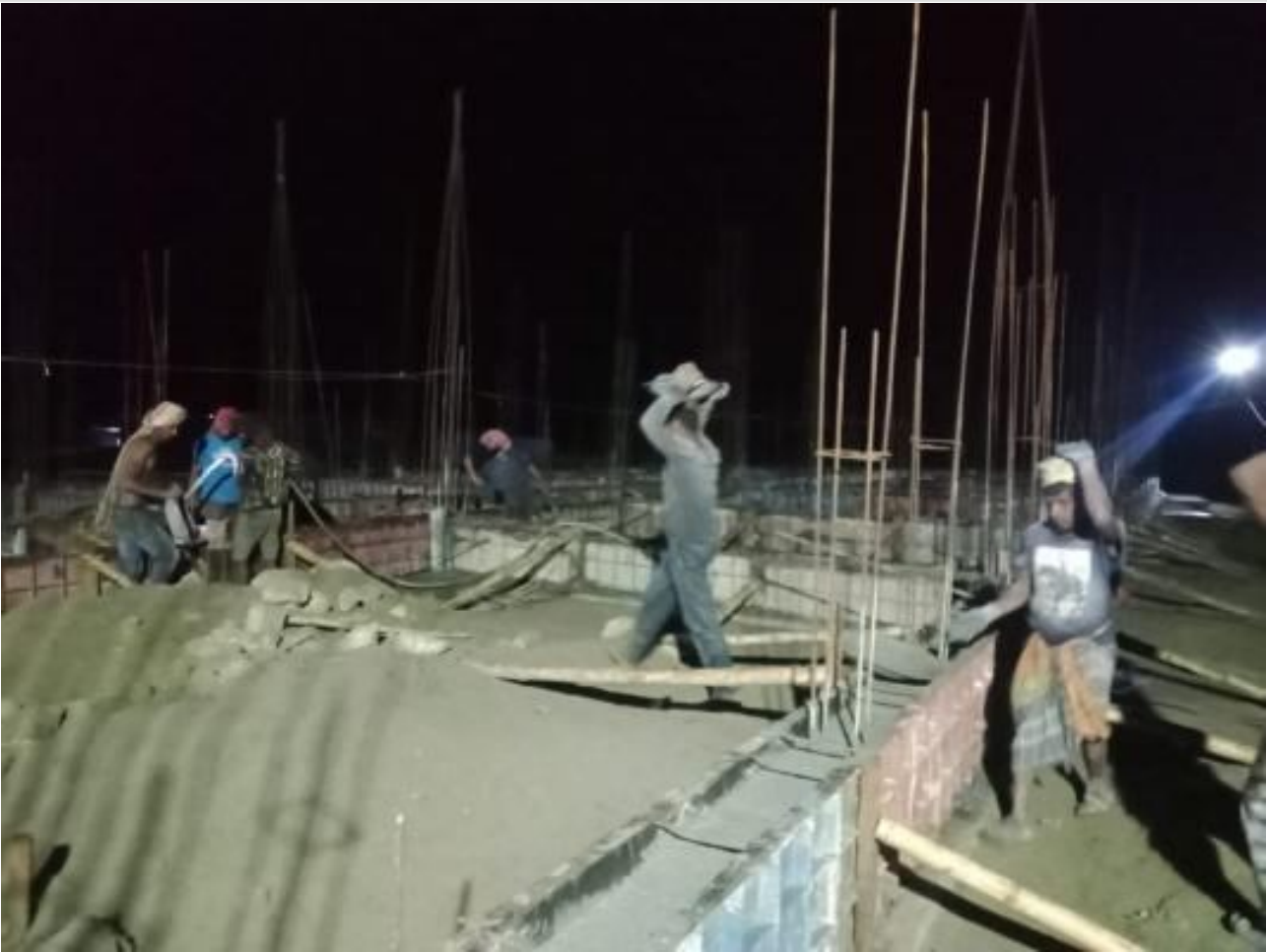
GB Concreting on 16-05-23
