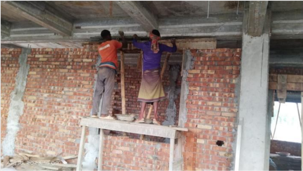
Comp-GF Brickwork on 18-08-23
