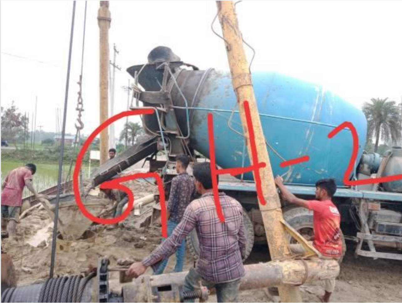
Guard House pile concreting by RMC on 19-03-23
