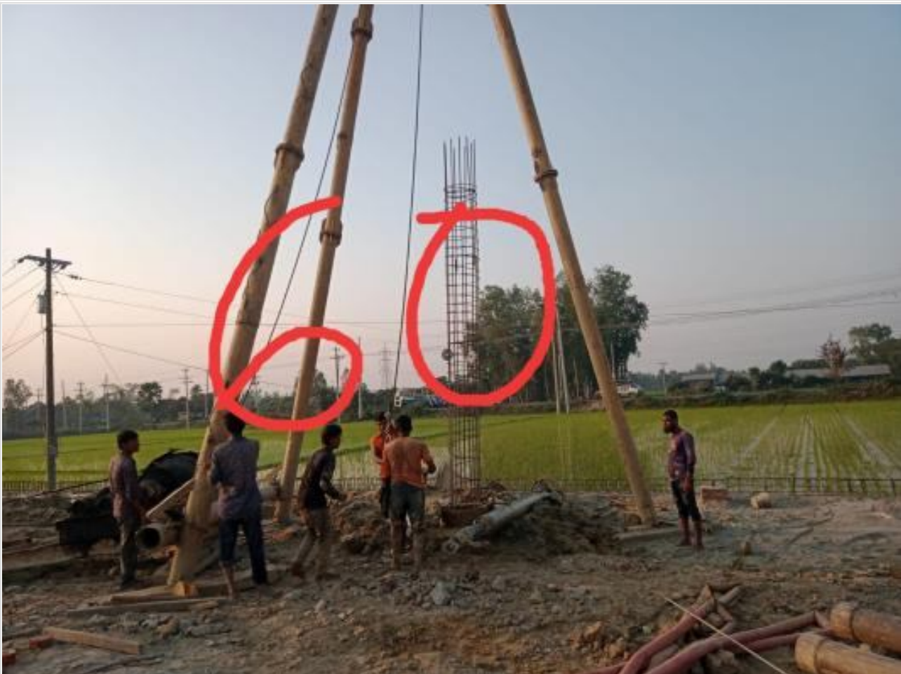
Ready mix concreting of pile on 12-03-23
