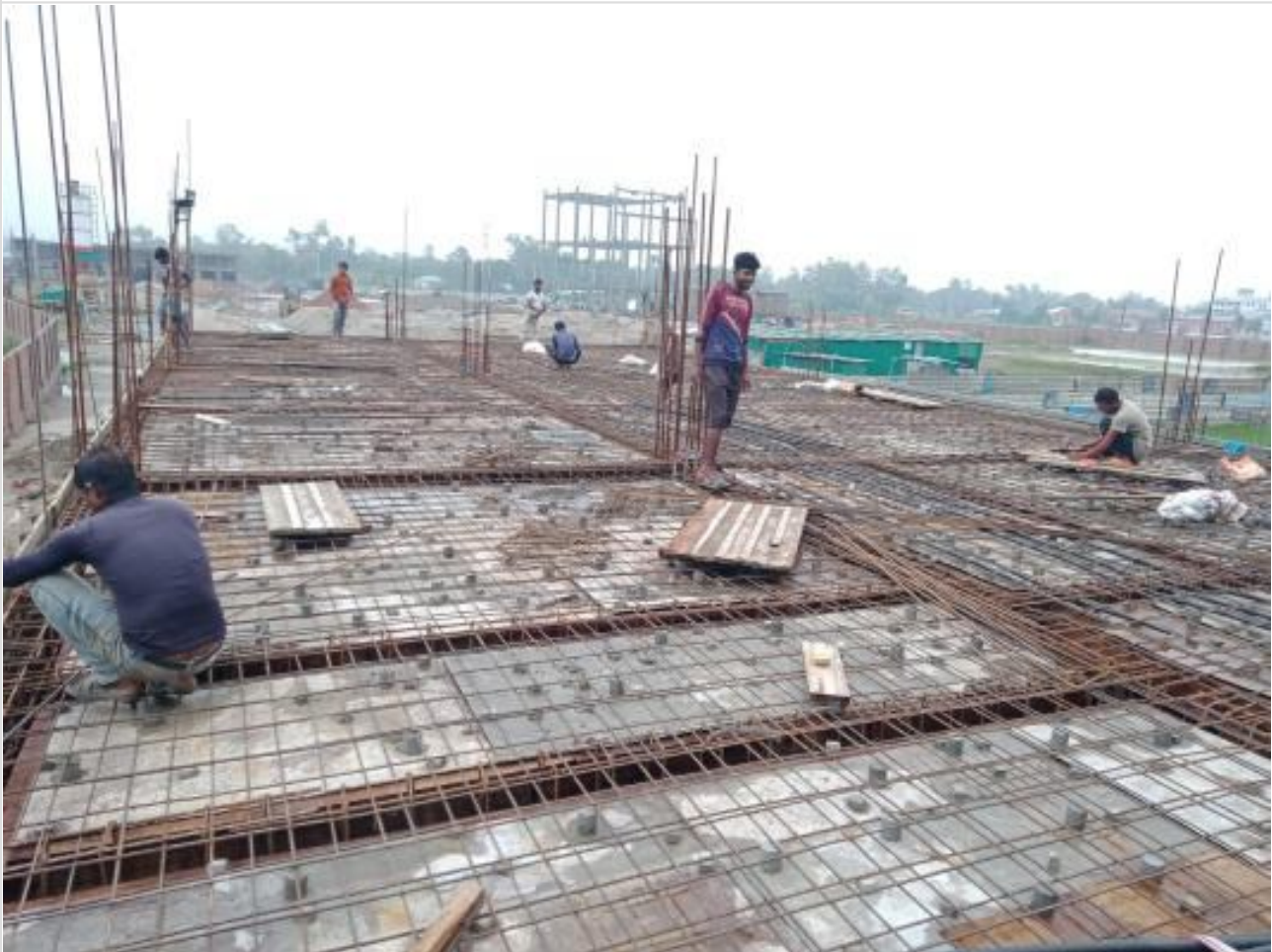
Dormitory Slab Electrical Pipe Laying on 08-08-23
