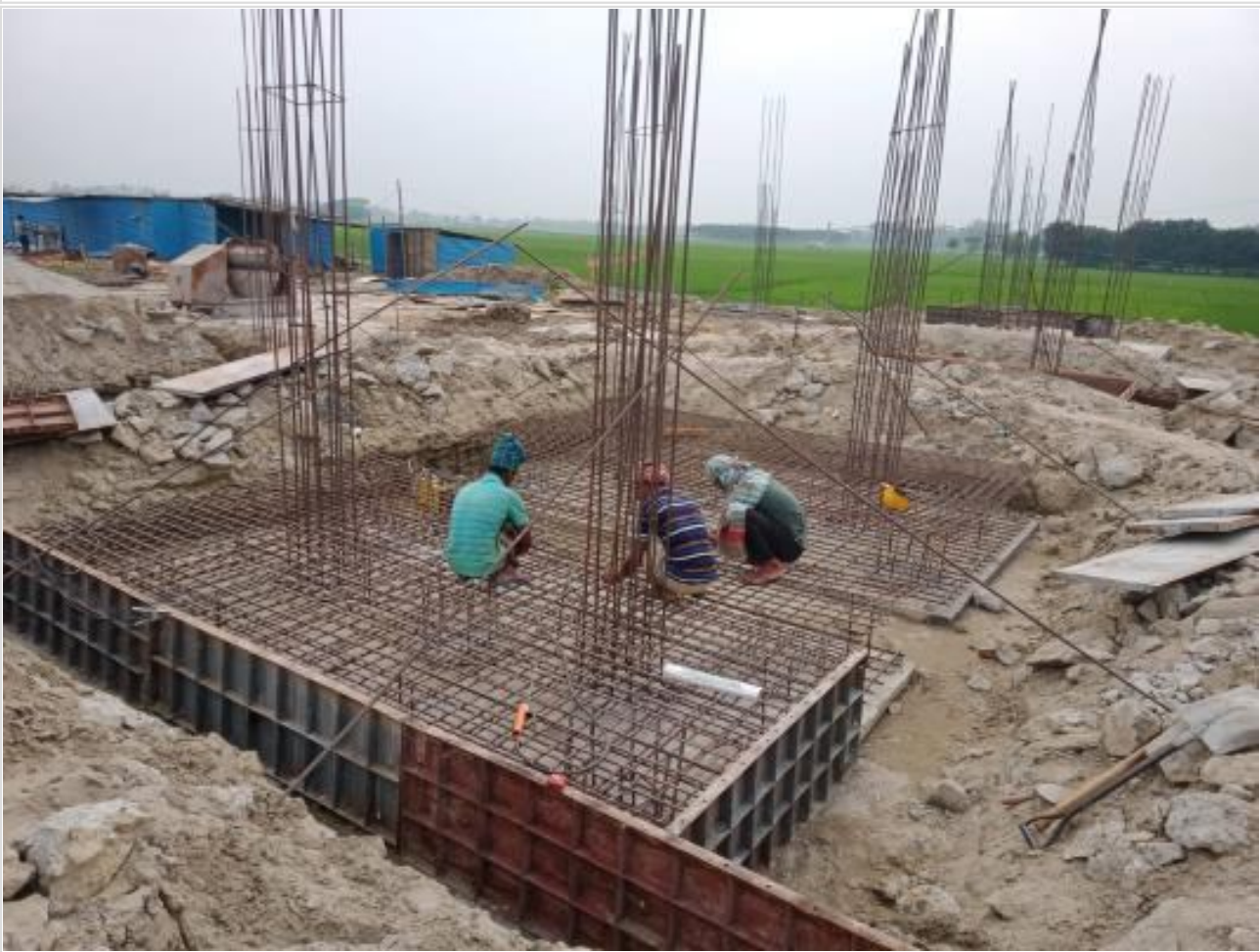
Pile Cap rebar binding on 15-04-23
