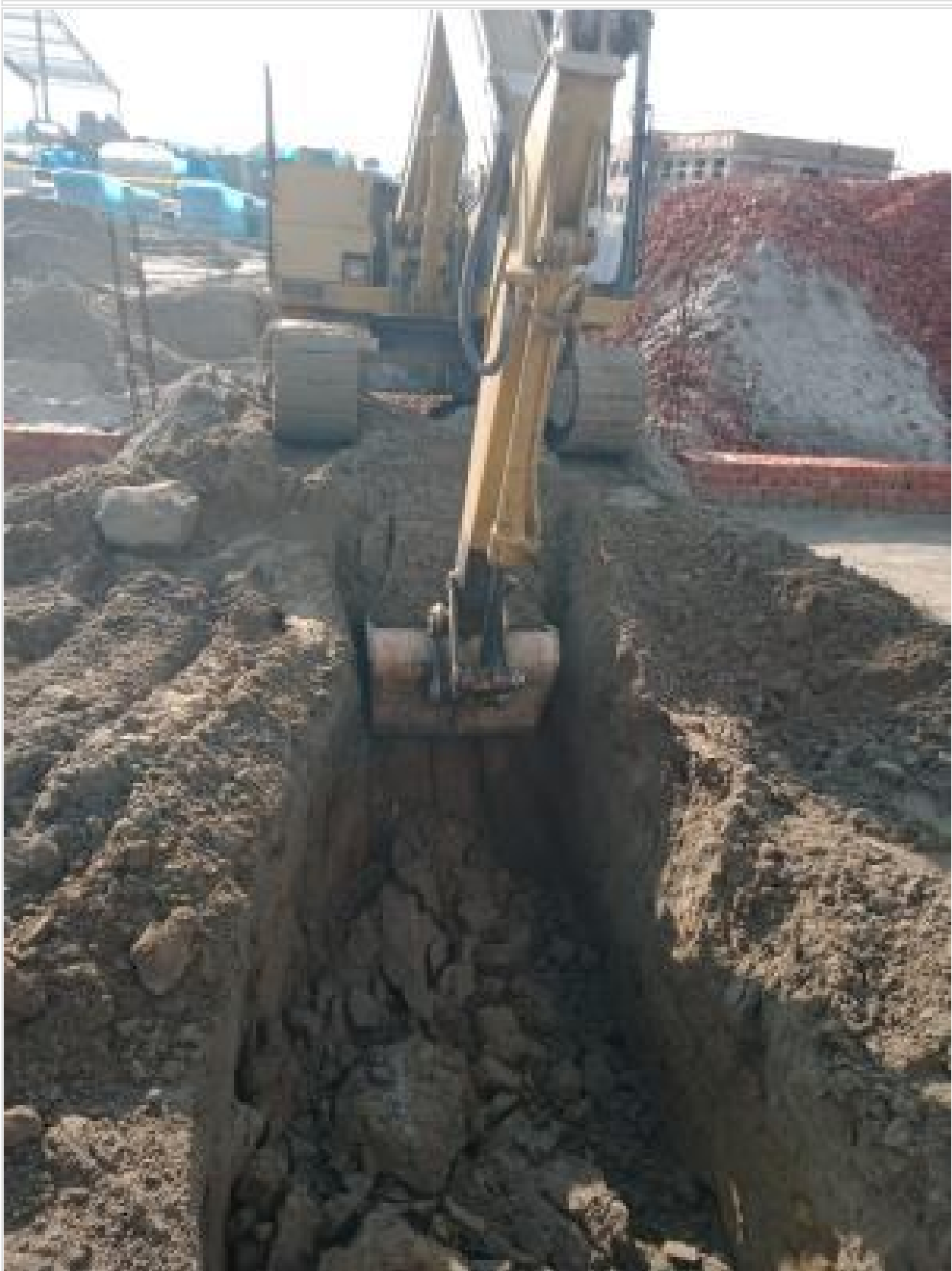
Earth cutting Electric line on 01-10-23
