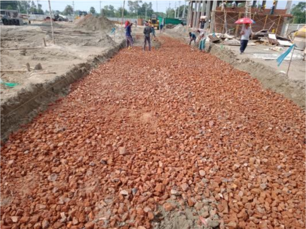
Road-Sub-base work on 21-08-23
