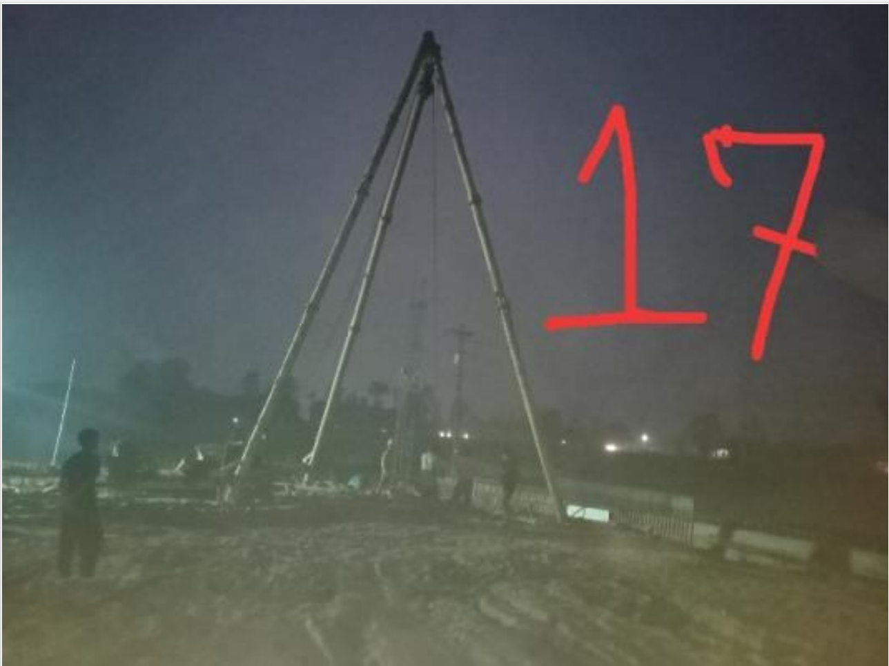
Com. Bldg. 17th Pile Boring on 21-02-23
