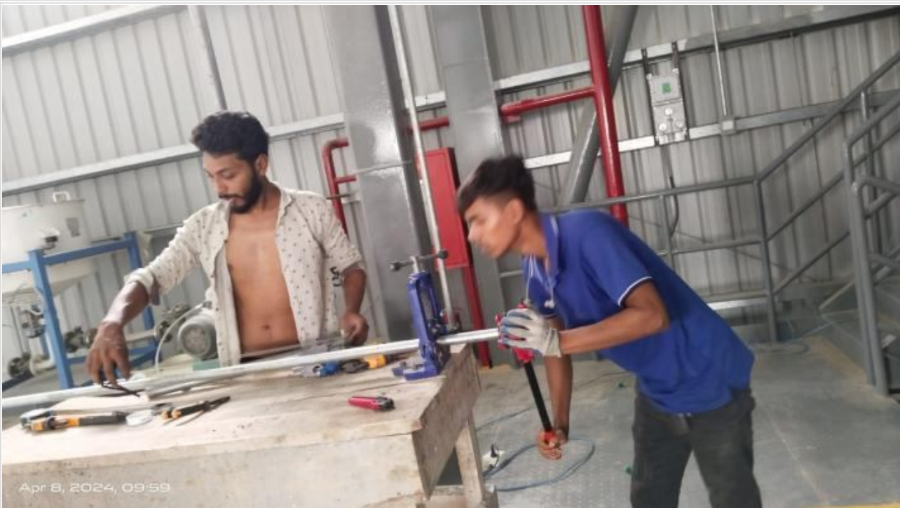
Electrical Work on 08-04-24
