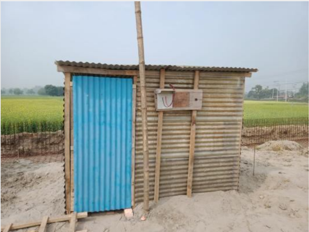
Electrical DB Setting on 31-01-23
