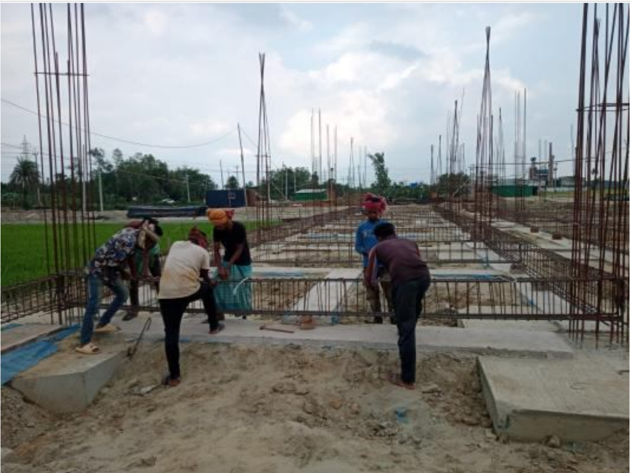
Re-bar work for GB of comp. Bldg. on 04-05-23
