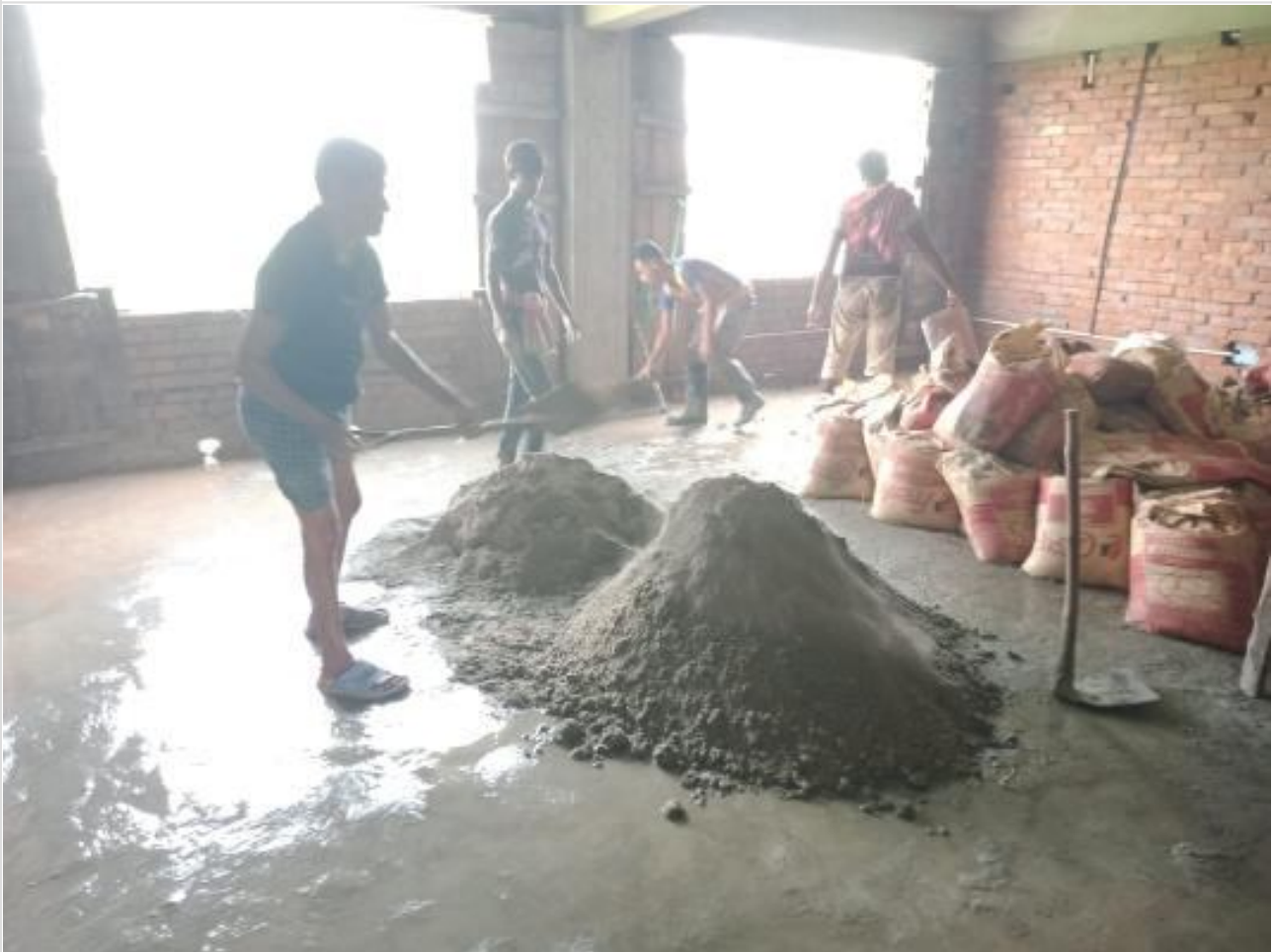
Comp. Bldg. GF casting on 29-09-23
