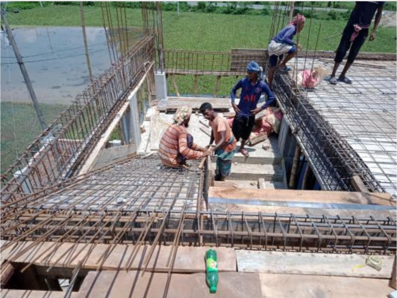
Comp. Bldg Rebar work on 31-07-23
