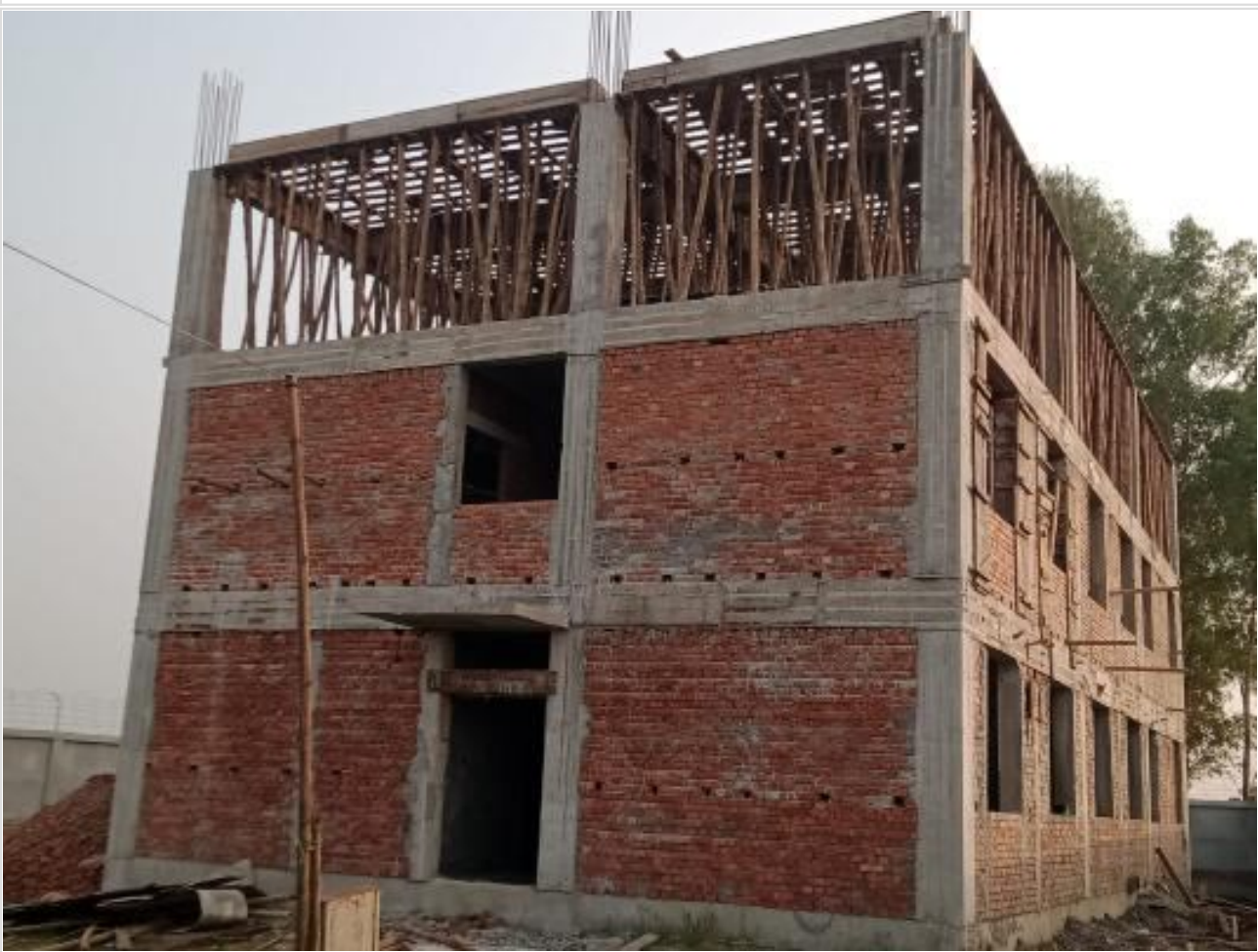
Dorm. Bldg. 3rd floor shuttering work on 09-11-23
