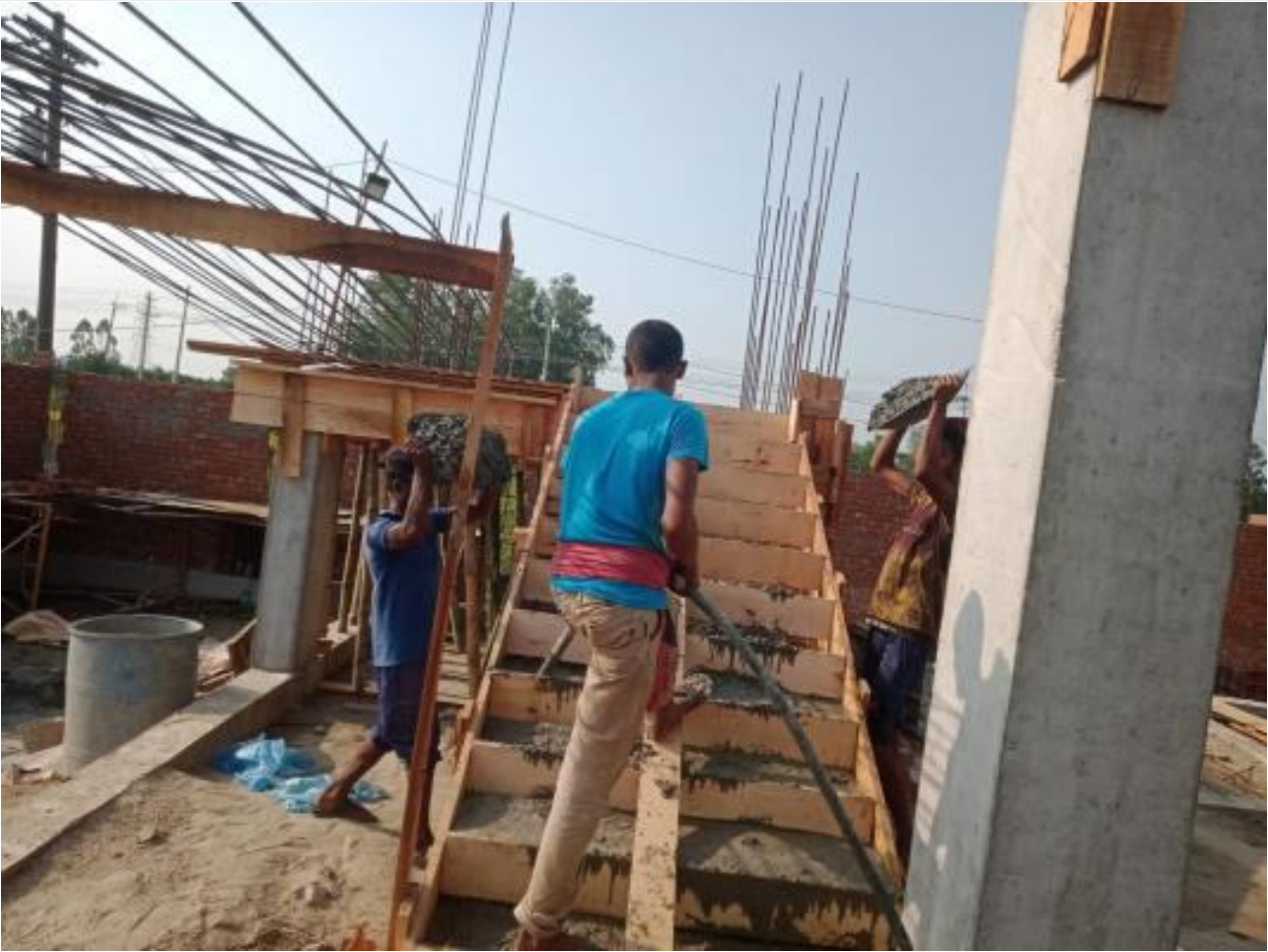
1st flight stair casting on 05-06-23
