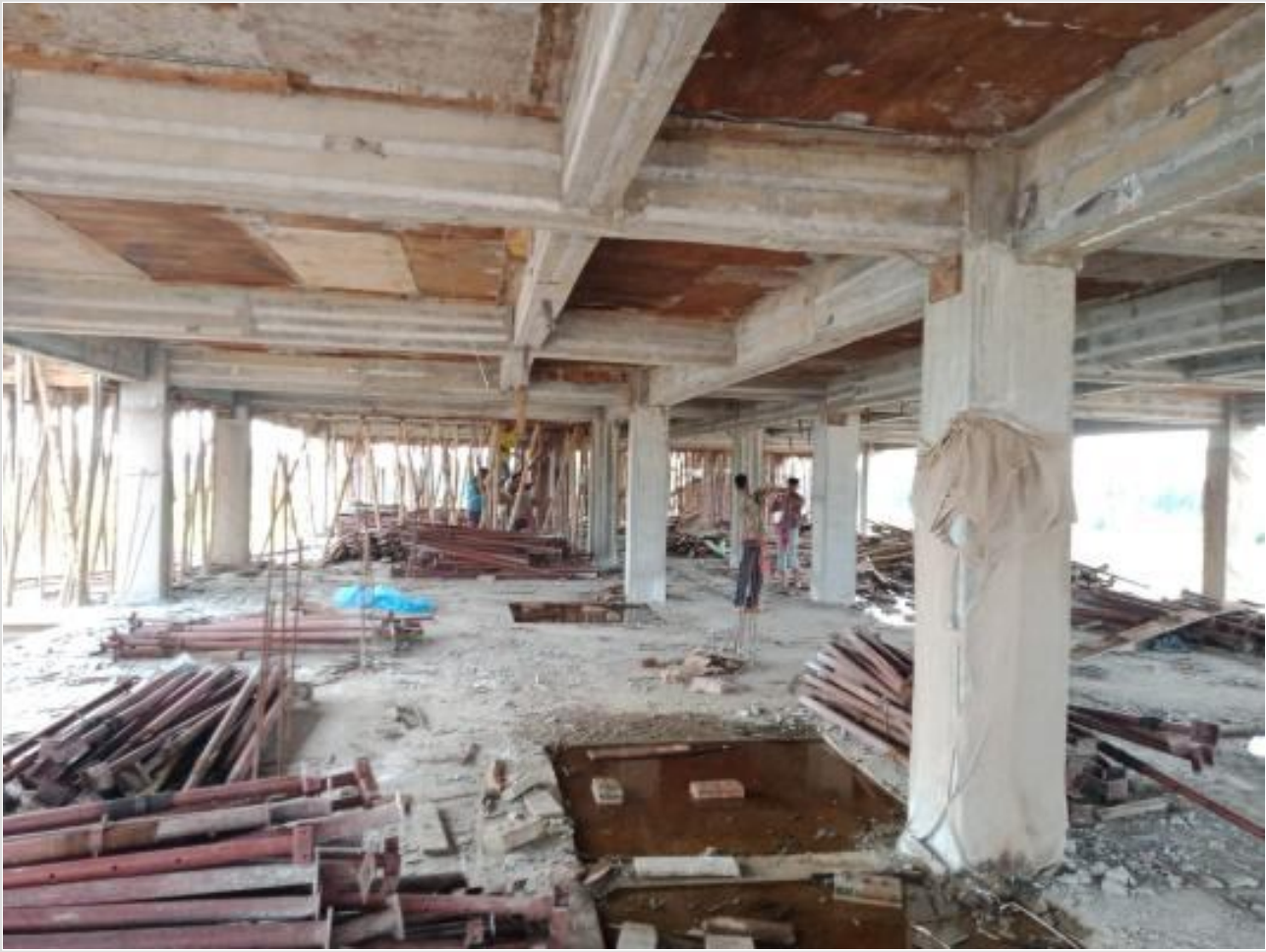
Comp-1st Floor-Shutter Removing on 20-08-23
