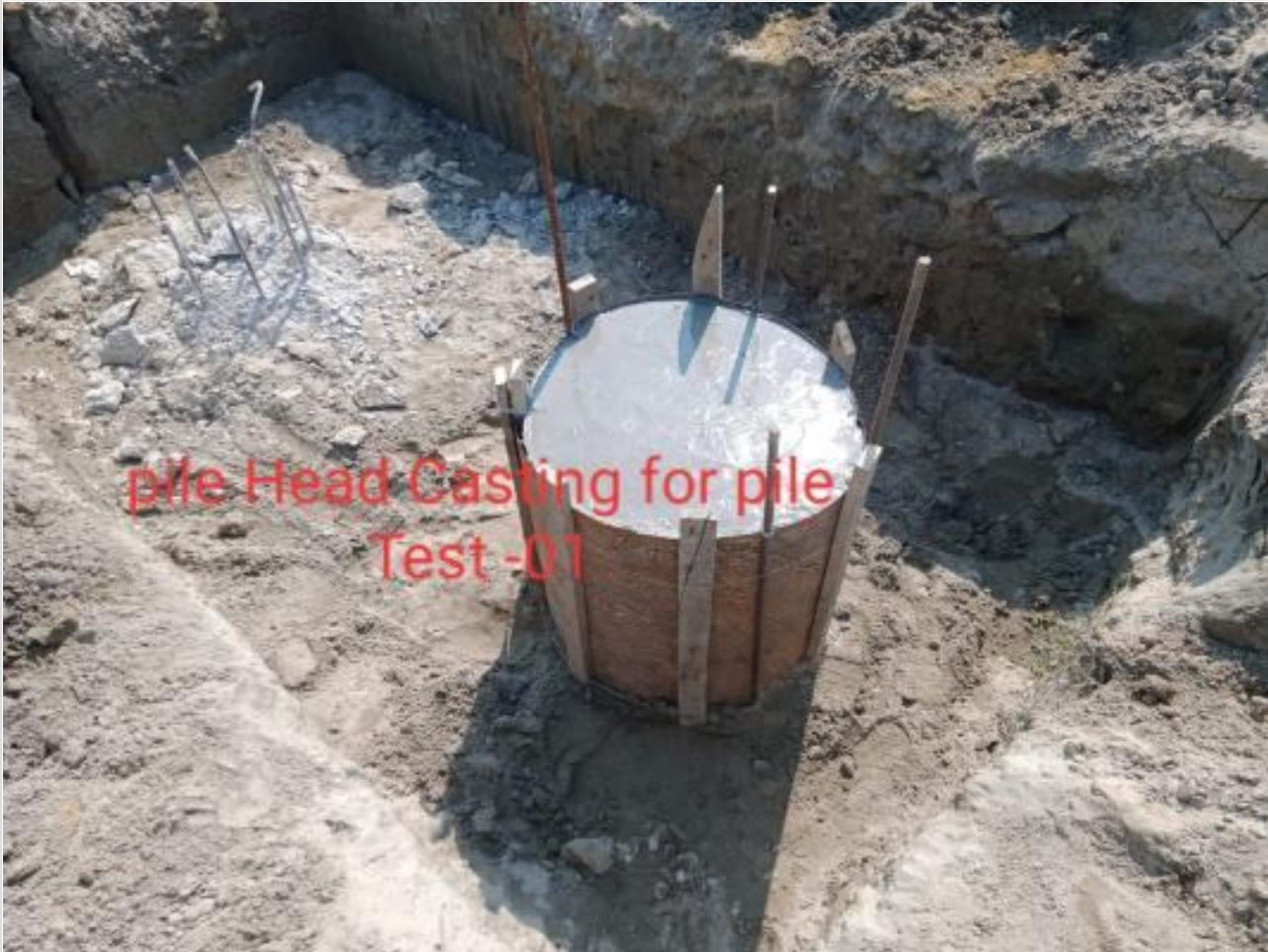
Pile head finishing for test on 03-04-23
