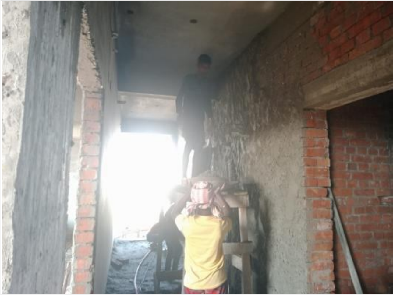
Dorm. Bldg. Plaster work on 02-11-23
