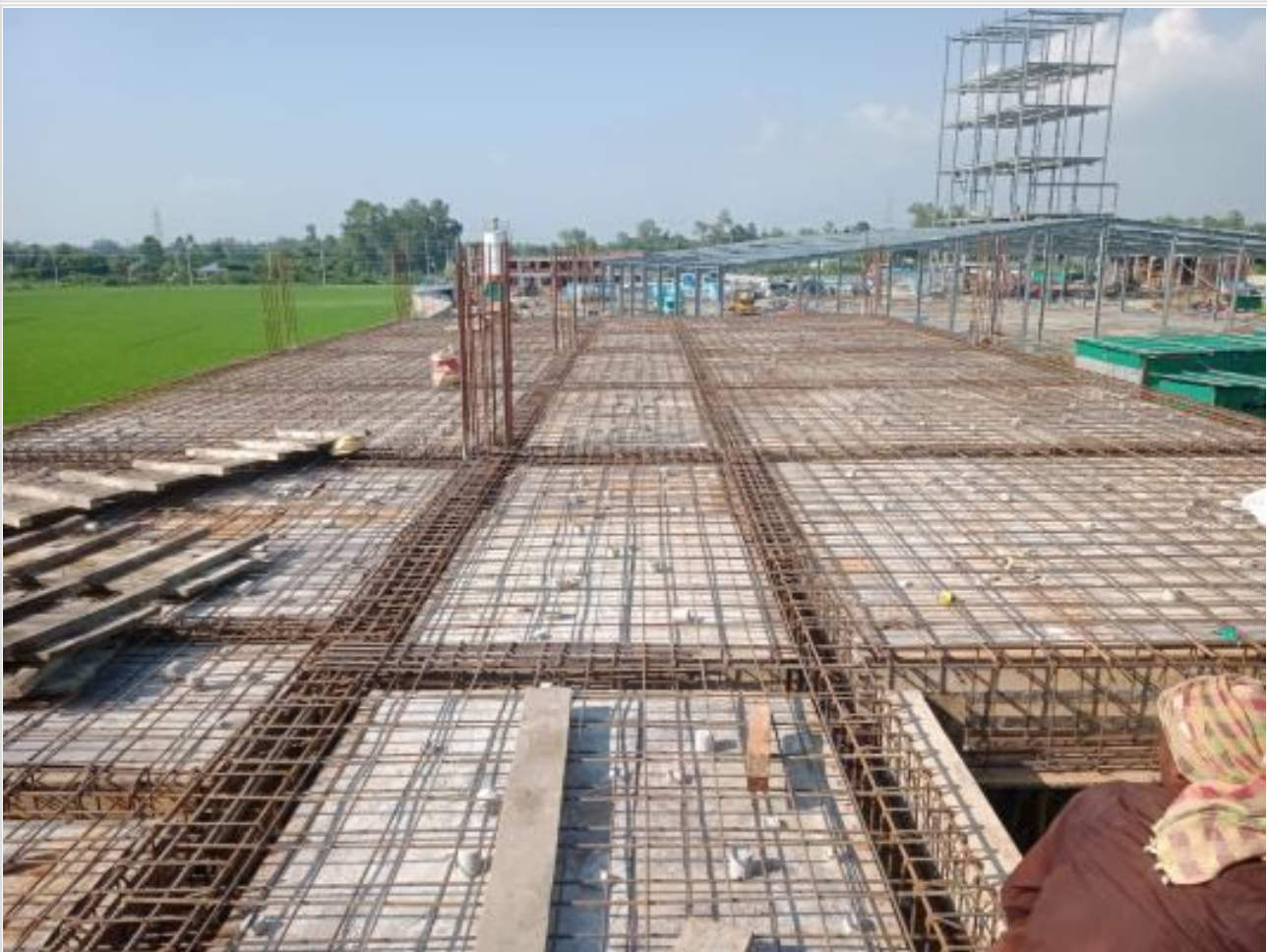
Dorm. Bldg. 2nd floor rebar work on 09-09-23
