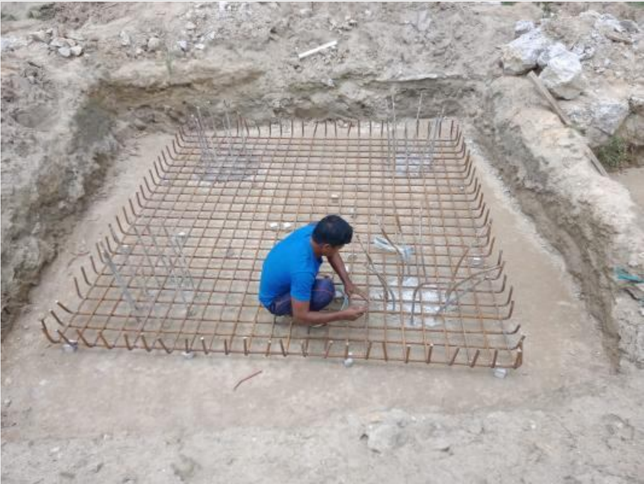
Dorm. Bldg. Pile cap rebar binding on 22-05-23
