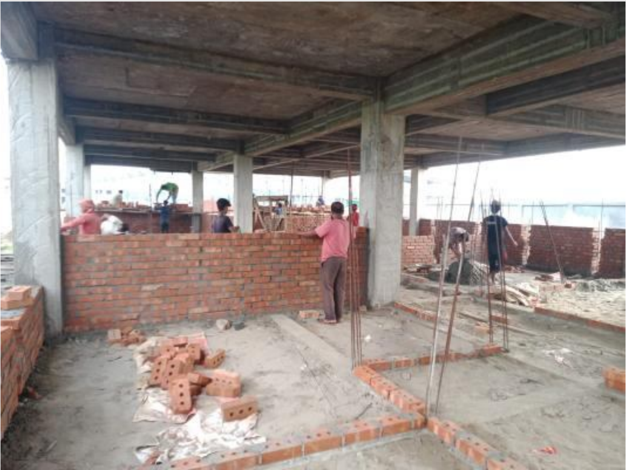
Dorm.Bldg brick work on 23-09-23
