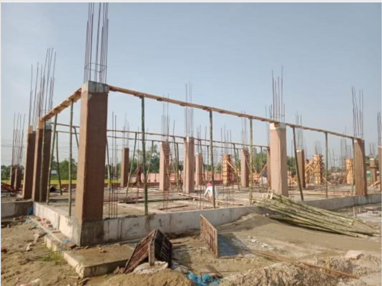
Comp. Bldg. Slab beam line shuttering on 01-06-23
