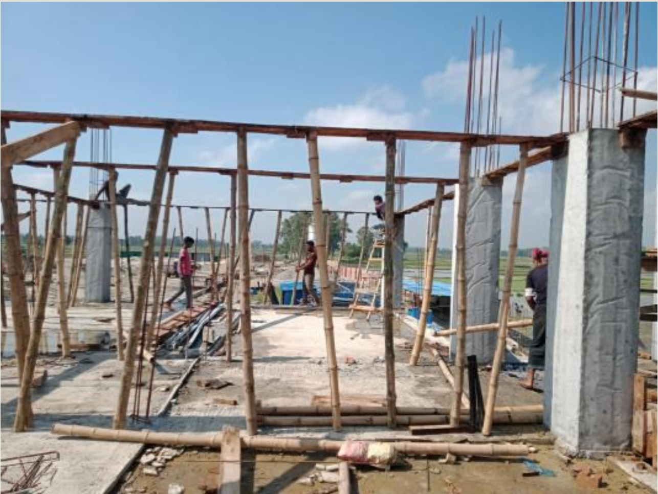
Comp. Bldg. 2nd Slab beam shuttering on 20-07-23
