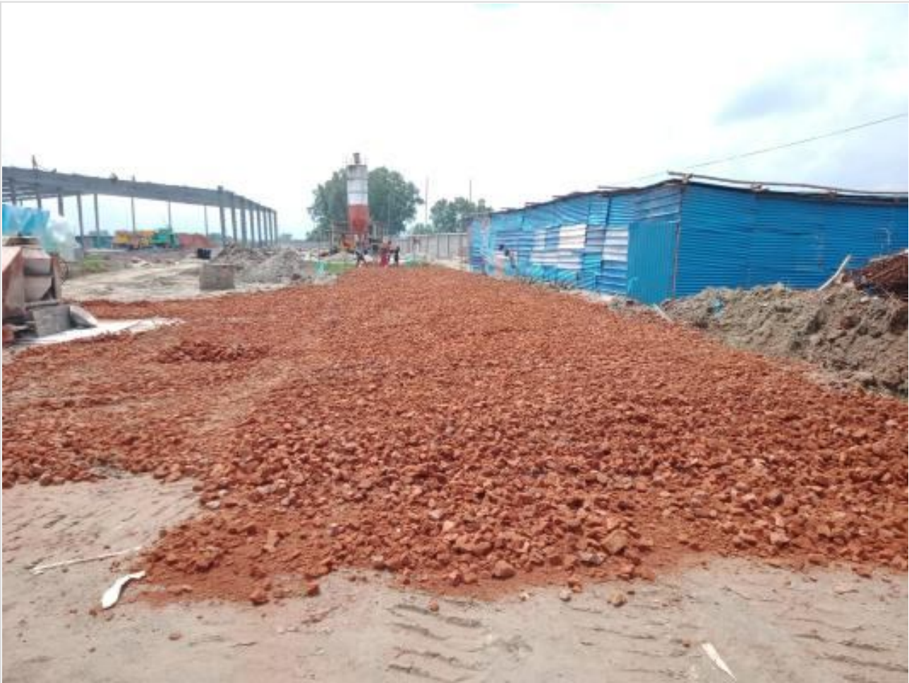
Road Sub-base work on 08-09-23
