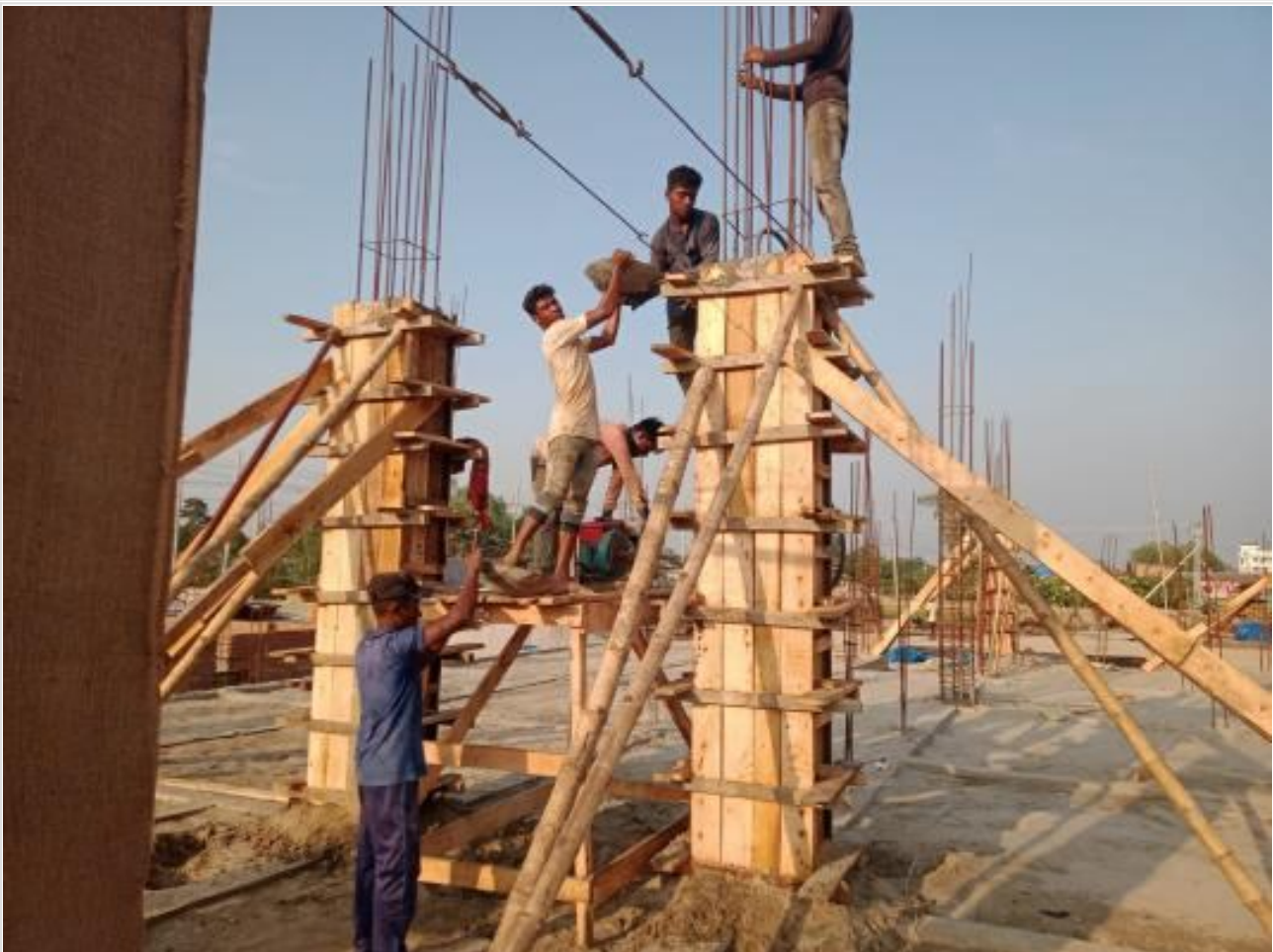
Comp. Bldg. Column casting on 30-05-23
