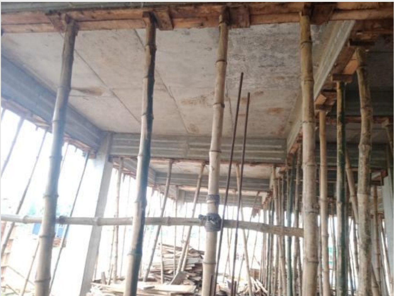
Comp. Bldg. Slab shutter opening on 12-07-23
