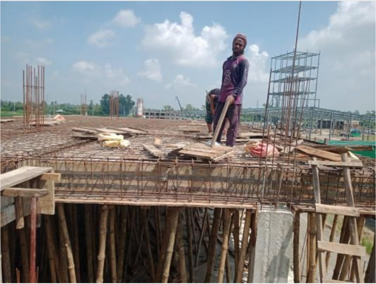
Comp. Bldg. FF Brick work on 10-09-23
