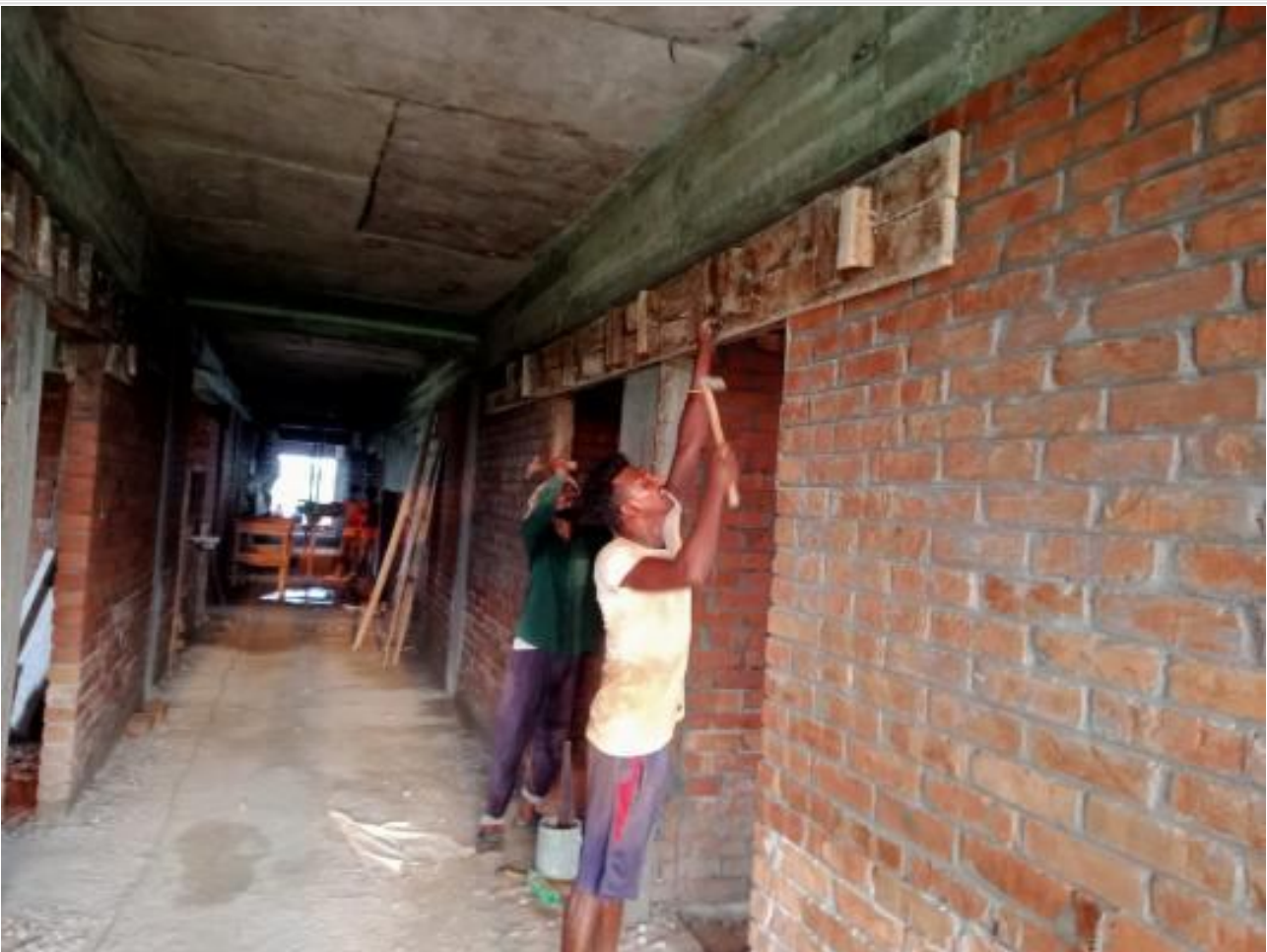
Comp. Bldg. Plaster work on 11-09-23
