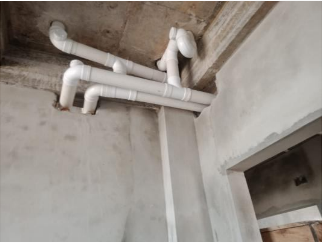
Comp. Bldg 1st floor sanitary work on 07-09-23
