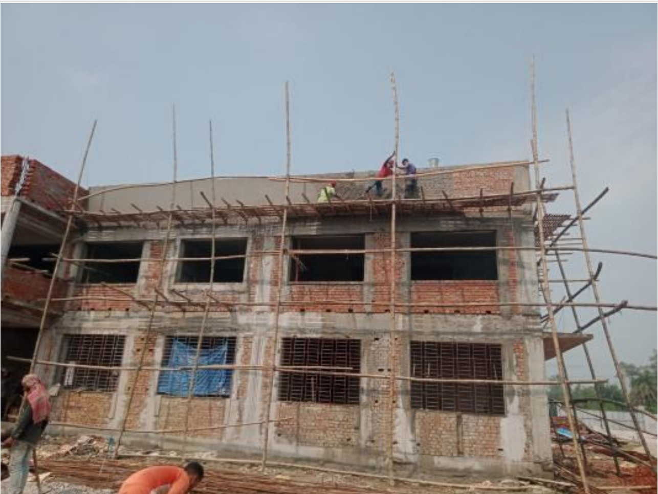
Comp. Bldg. Outside plaster work on 09-10-23
