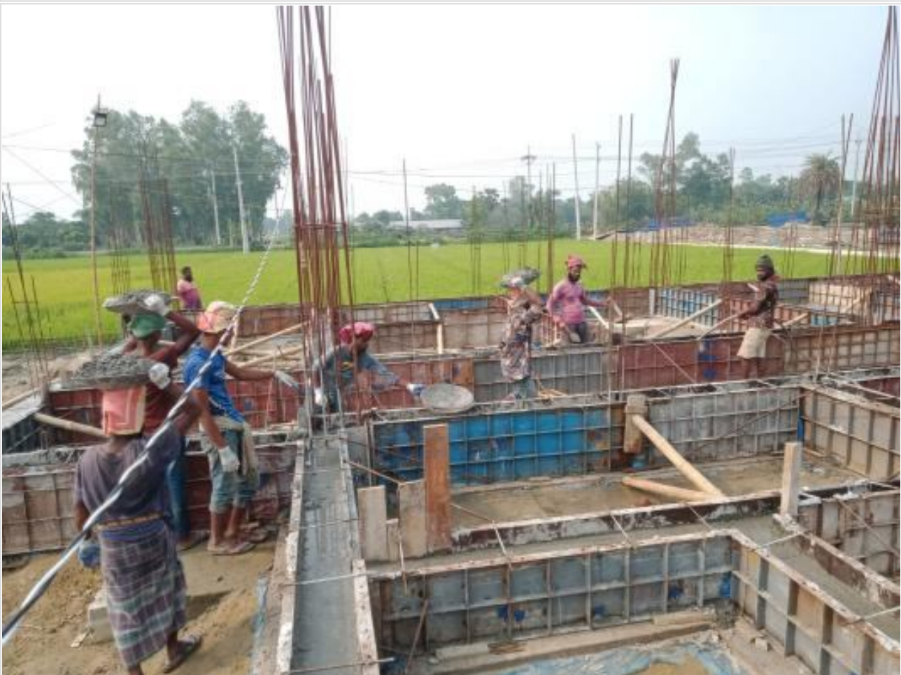
Comp. Bldg. GB casting work on 12-05-23
