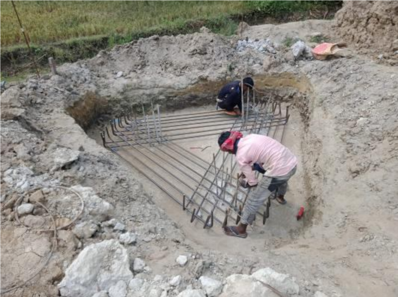
Dorm Bldg pile cap rebar binding on 23-05-23
