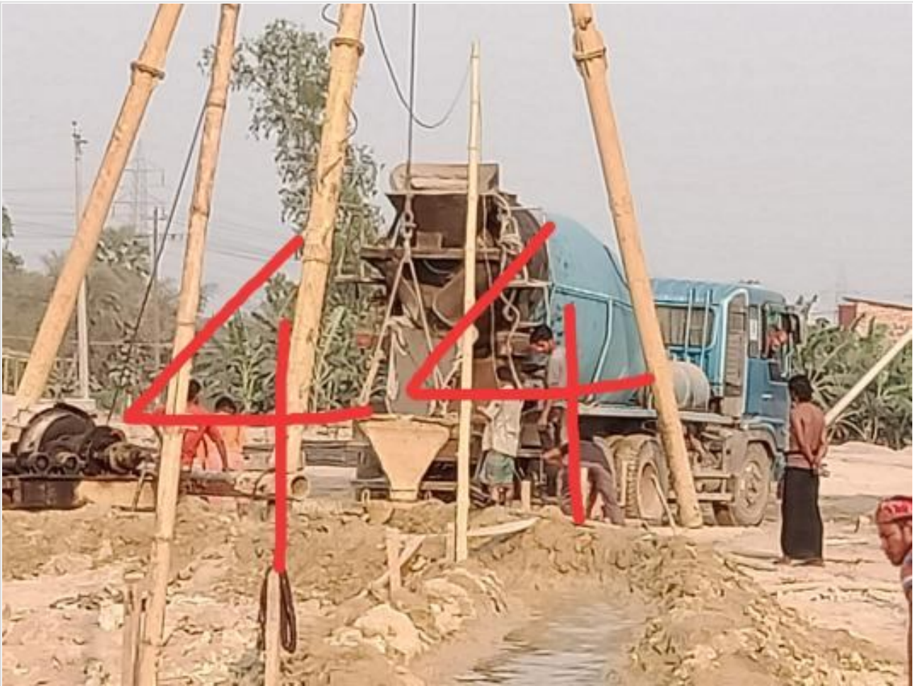
Ready mix concreting of pile on 05-03-23
