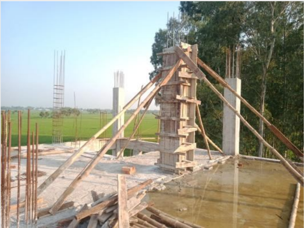
Dorm. Bldg. Roof top Column work on 13-10-23
