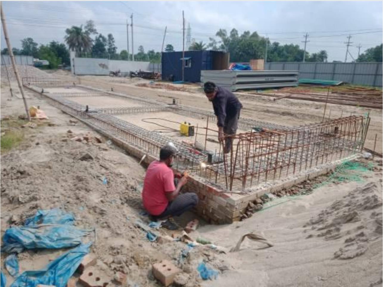
Anchor bolt fitting at scale on 06-09-23
