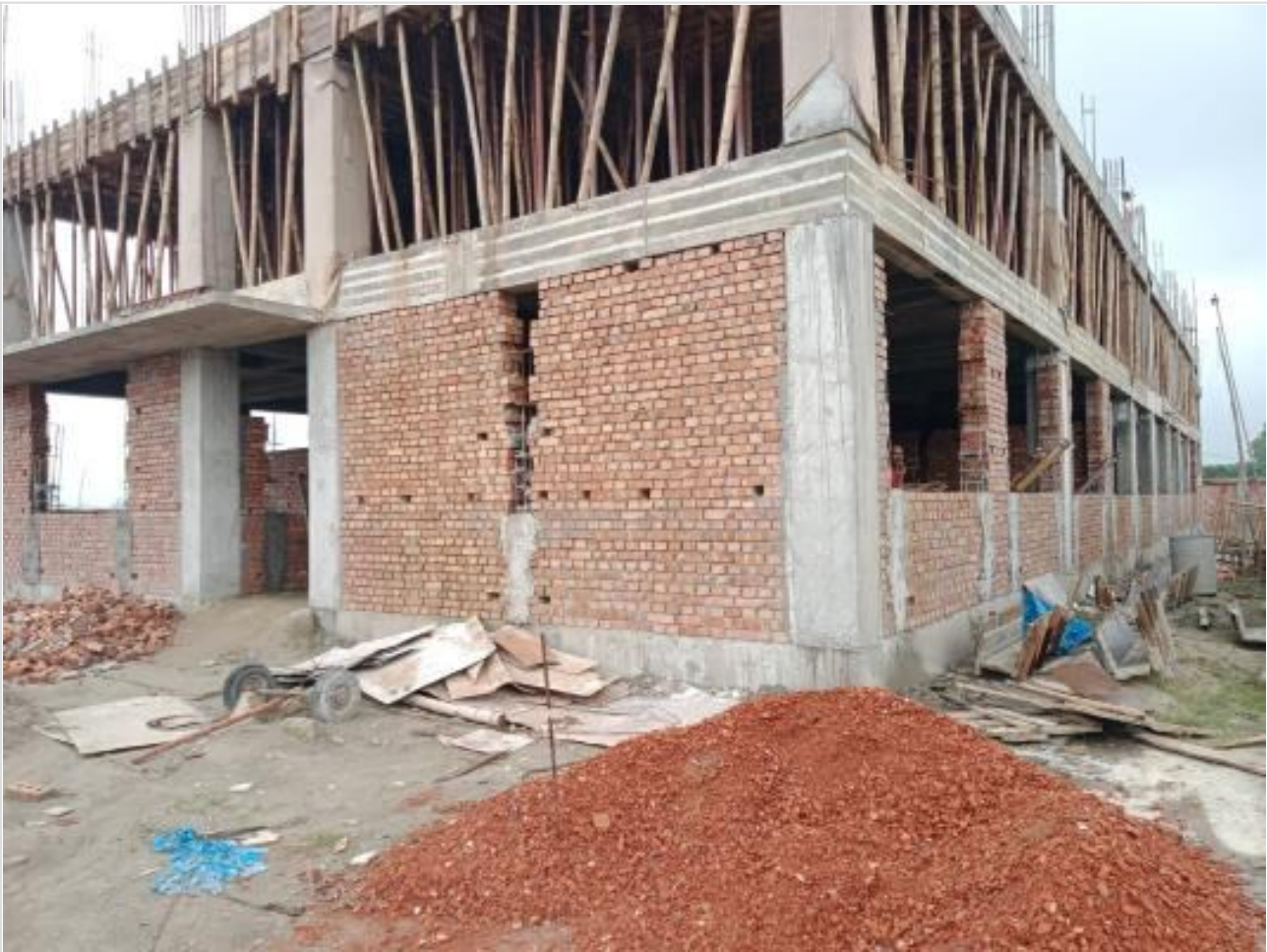
Comp.Bldg GF Brick work on 06-08-23
