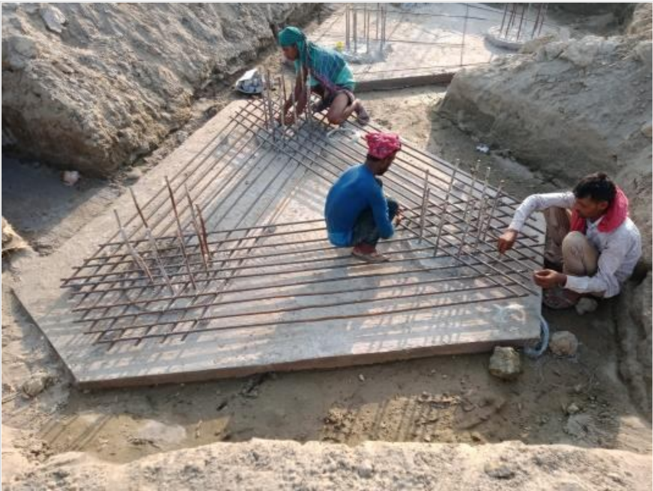
Pile cap work on 14-04-23
