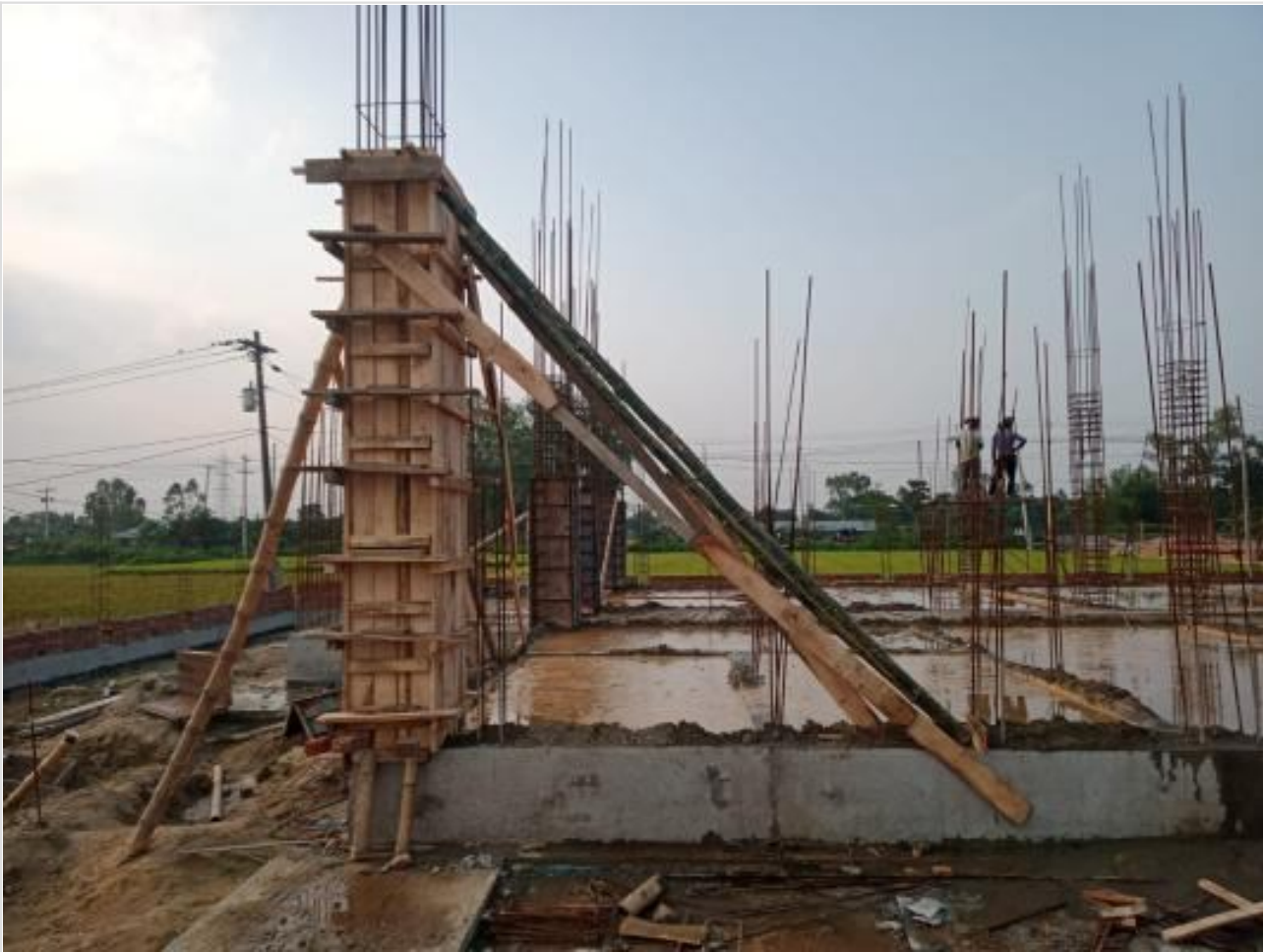
Comp. Bldg column shuttering on 26-05-23
