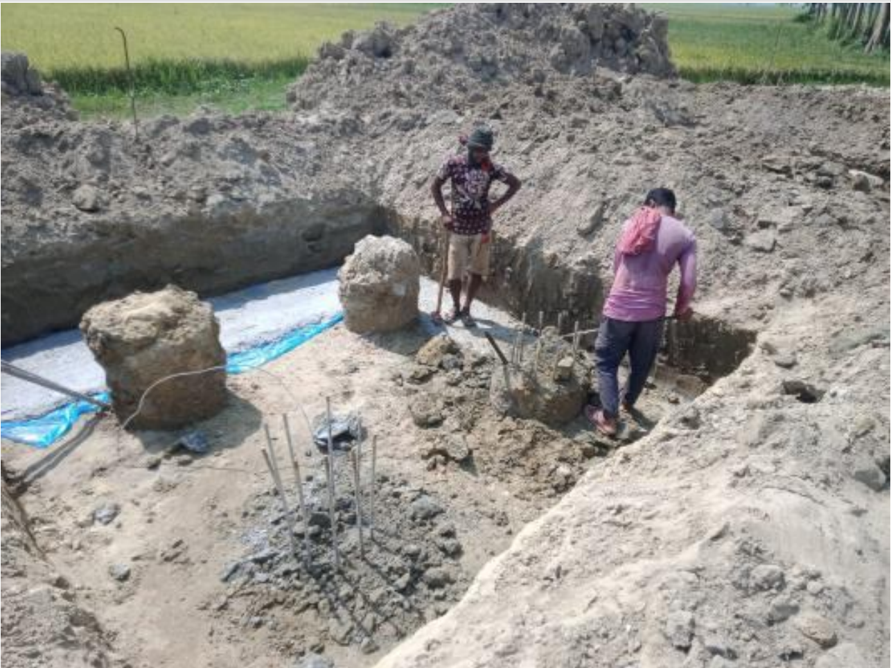
Dorm. Bldg. pile head breaking on 10-05-23
