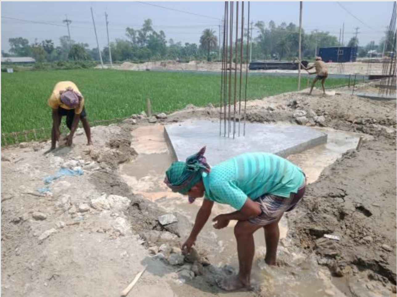
Back filling and levelling dressing. on 19-04-23
