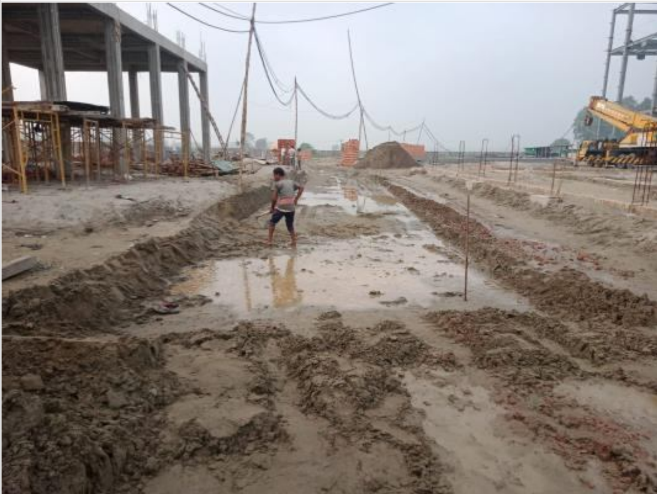
Road-Excavation-box cutting on 16-08-23
