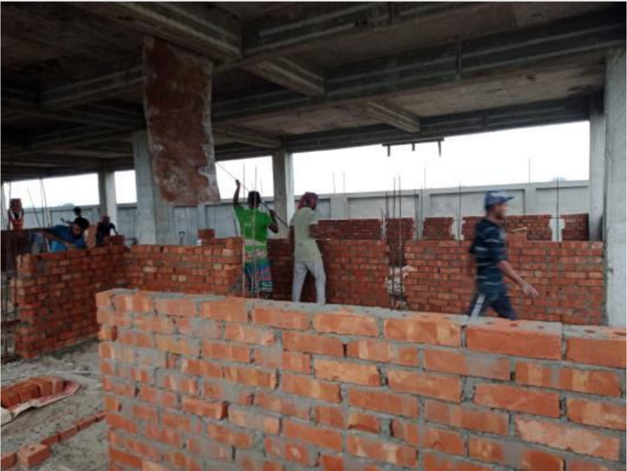
Dorm. Brick work on 22-09-23
