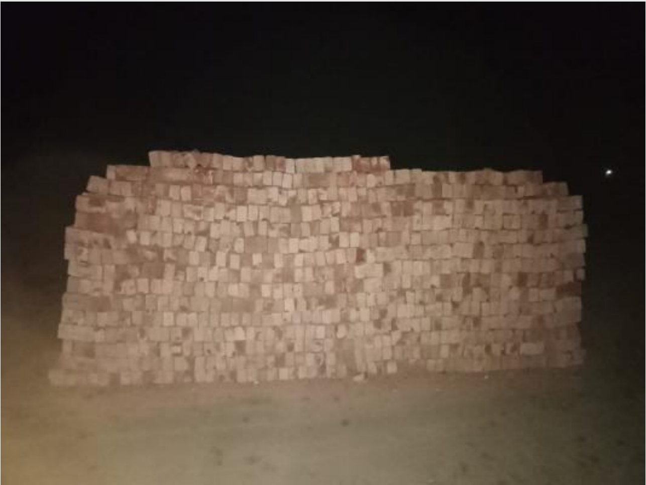
Brick mobilized for shed on 09-01-23
