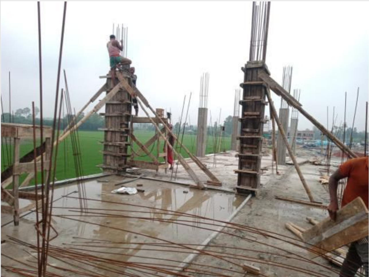
Dormitory bldg. Column casting on 26-08-23
