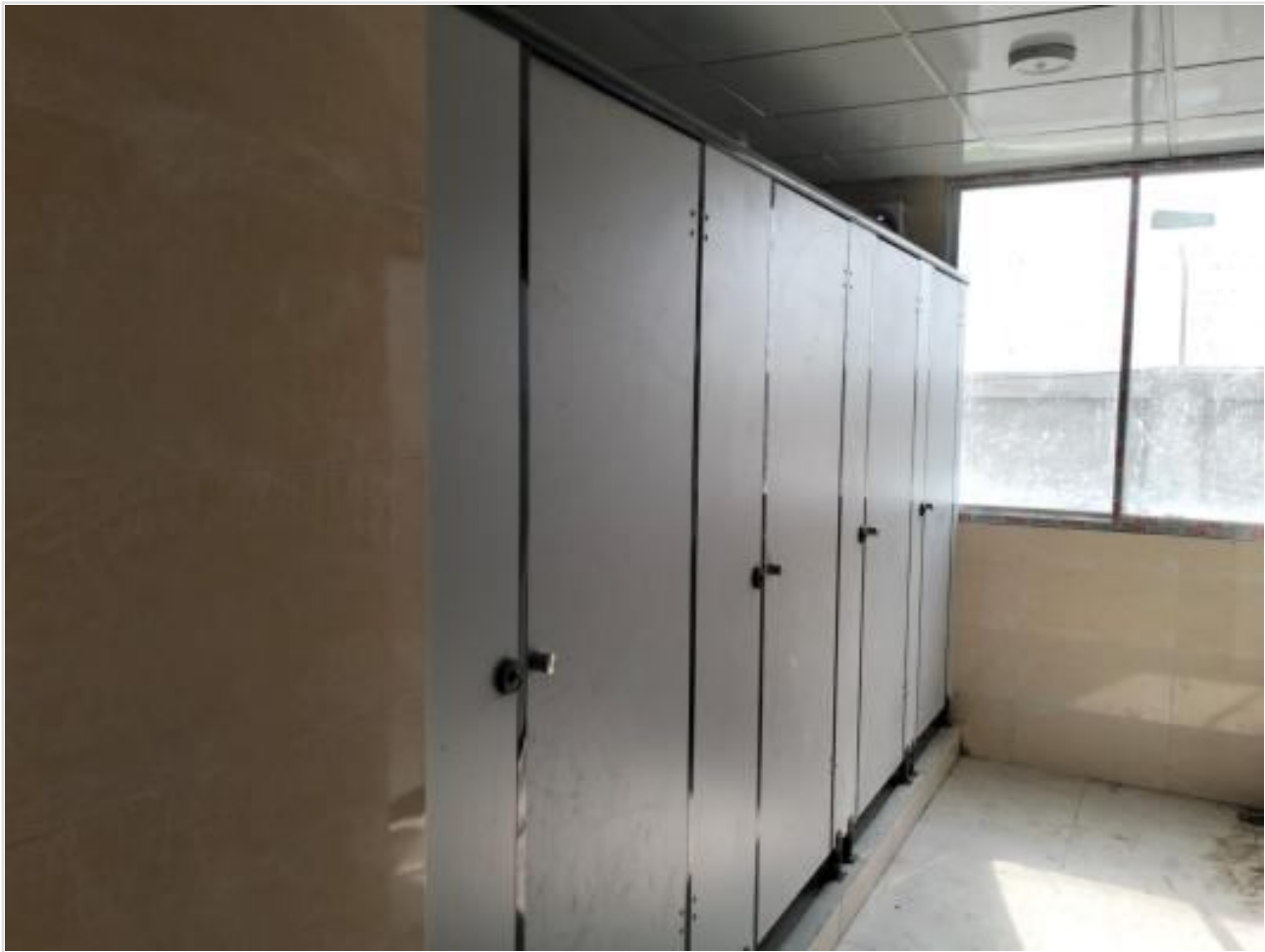
Dormitory-Inside-Toilet Area on 26-02-24
