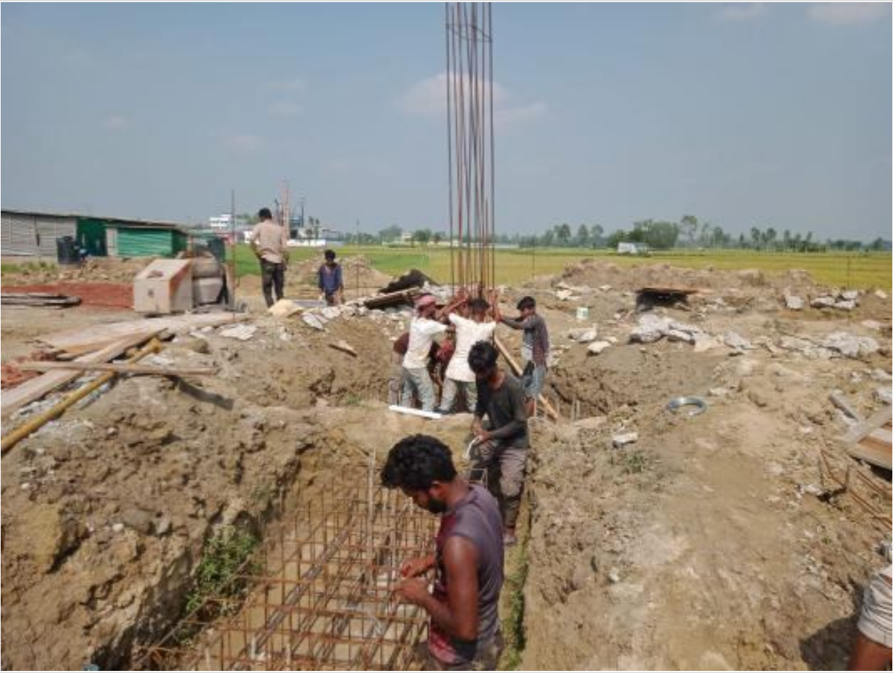
Dorm. Bldg. Pile cap rebar binding on 24-05-23
