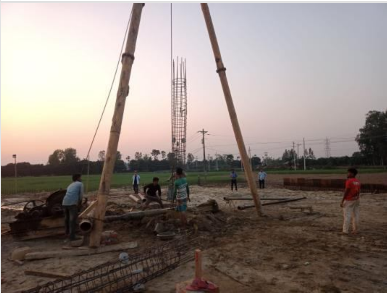
Pile boring work on 14-02-23
