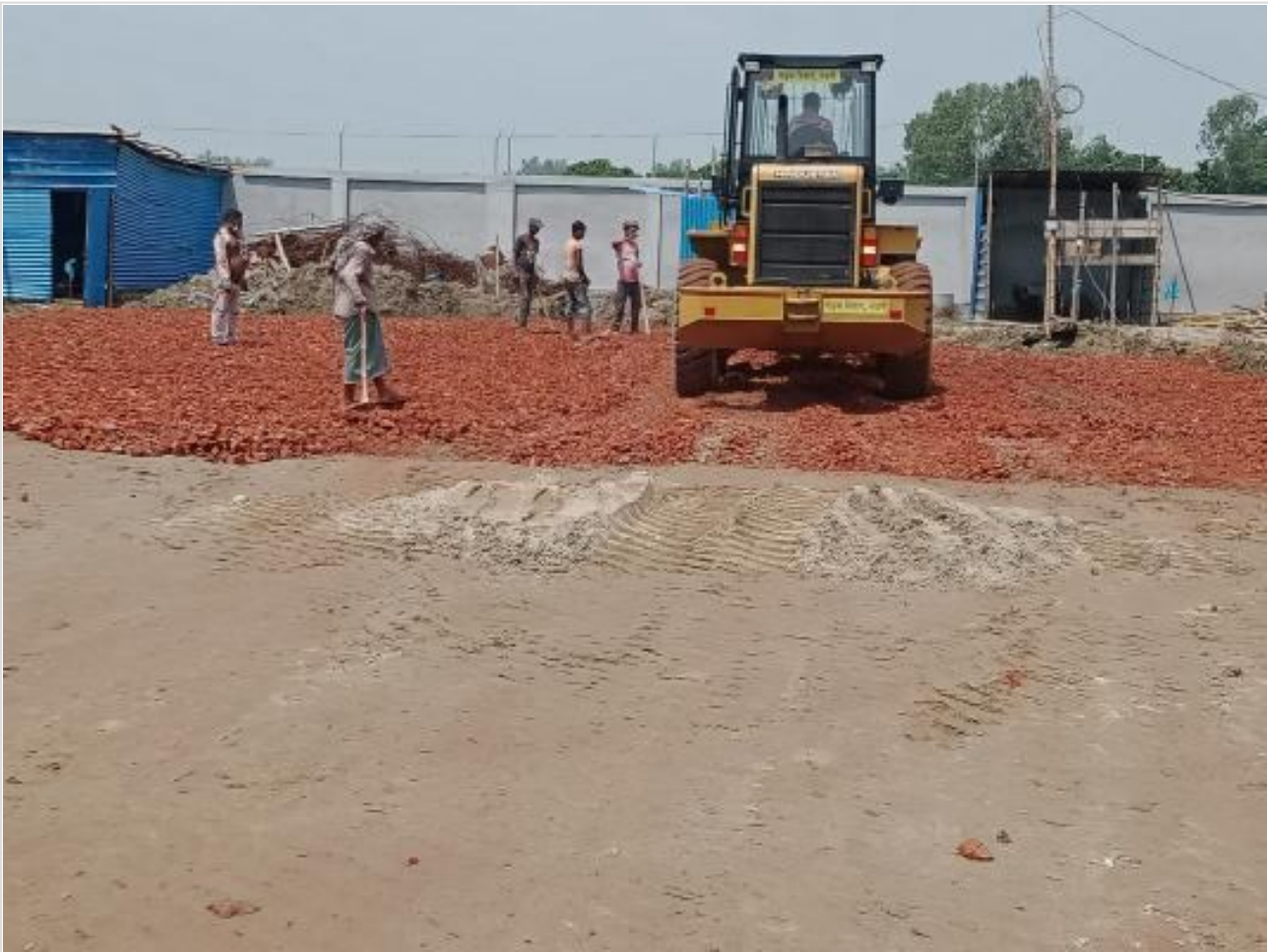
Road Sub-base work on 30-08-23
