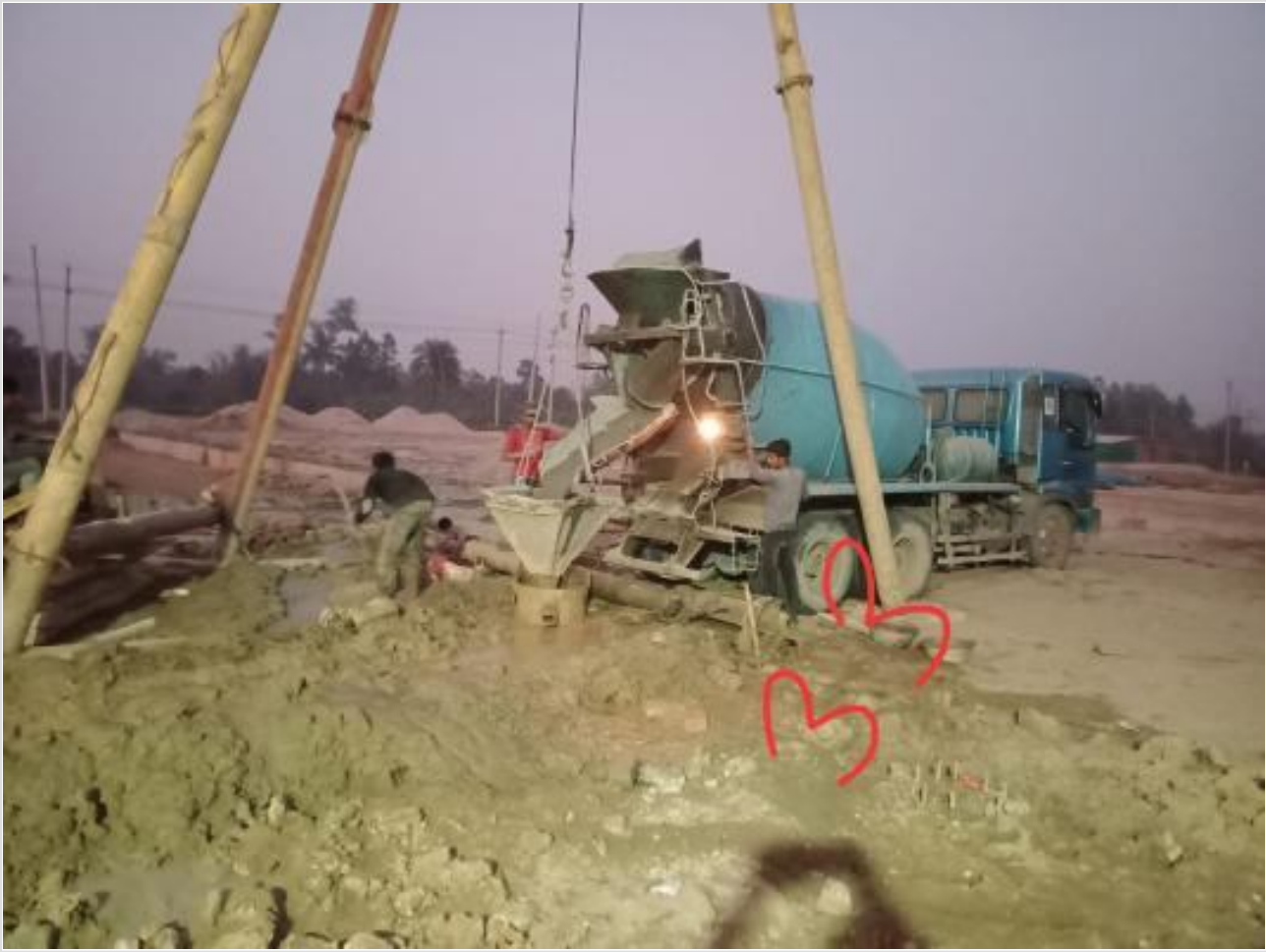
Ready mix concreting of pile on 27-02-23
