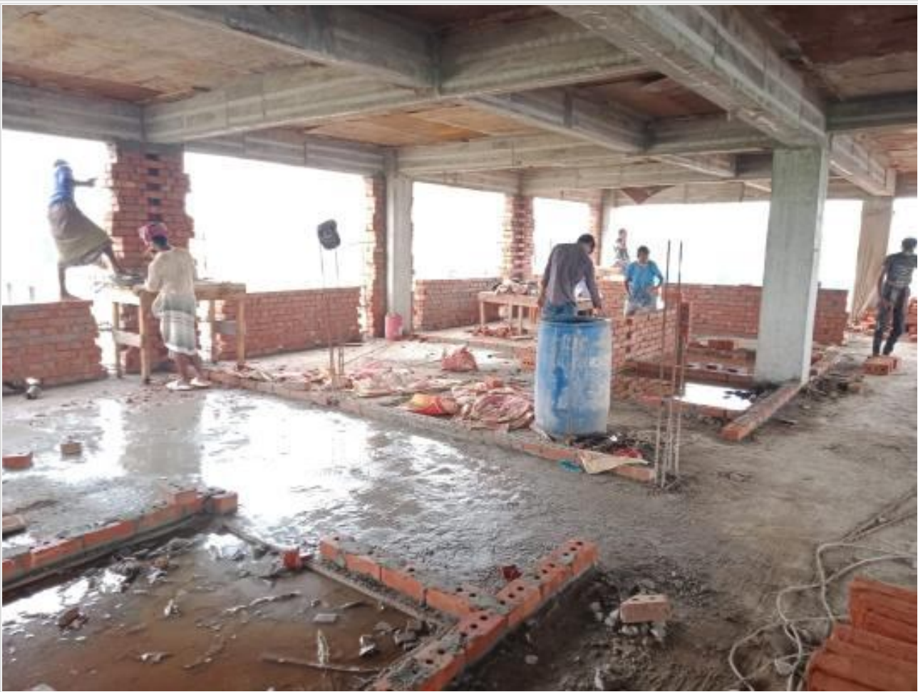
Comp. Bldg. 1st floor brick wall on 24-08-23
