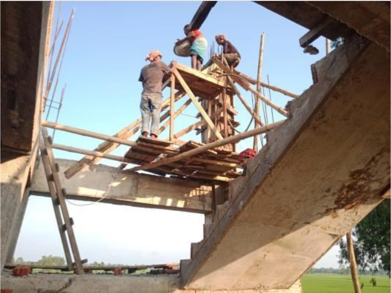
Dorm. Bldg. Roof top column casting on 08-10-23
