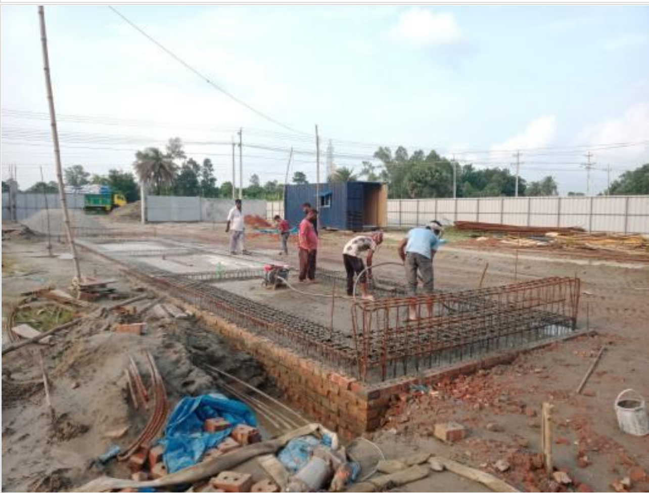
Weighing Bridge Concreting on 23-08-23
