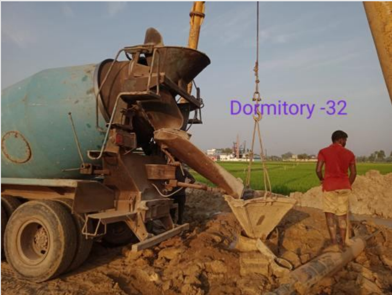
Dorm. Bldg. 32nd pile concreting on 09-04-23
