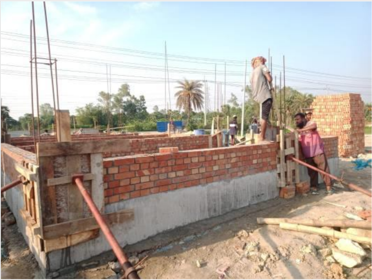
Gate house Brick work on 30-05-23
