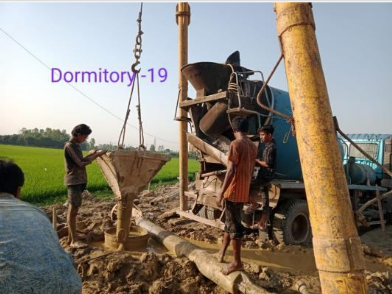
Pile cap bottom cc casting. on 04-04-23
