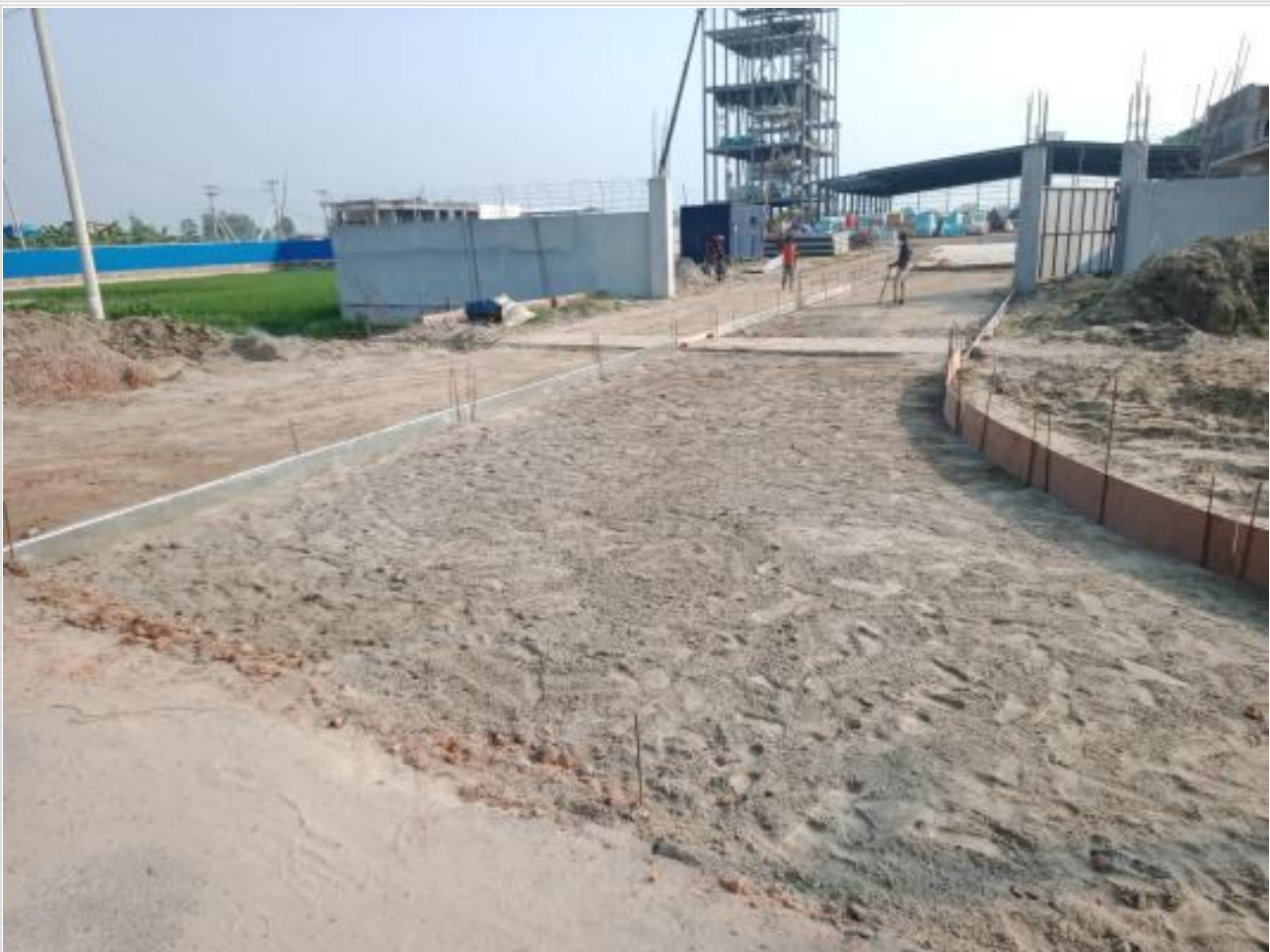
Road work on 14-10-23
