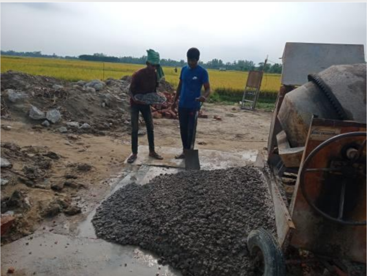
Dorm Bldg pile cap bottom cc casting on 17-05-23
