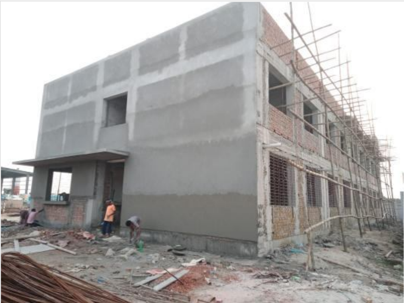
Comp. Bldg. Outside plaster work on 15-10-23
