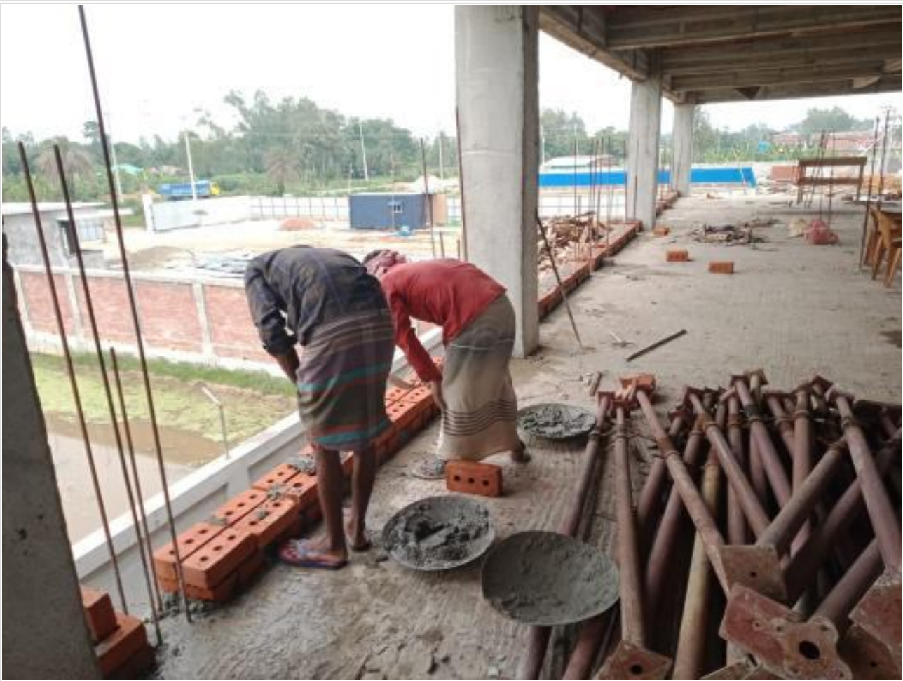
Comp-1st Floor-Brickwork on 22-08-23
