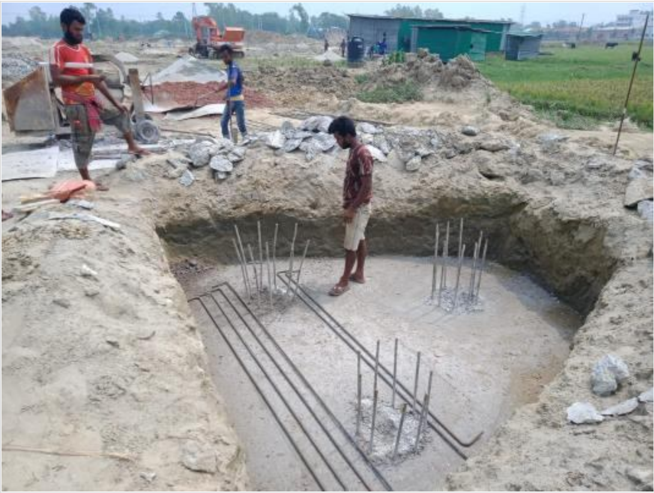
Pile cap rebar work on 23-05-23
