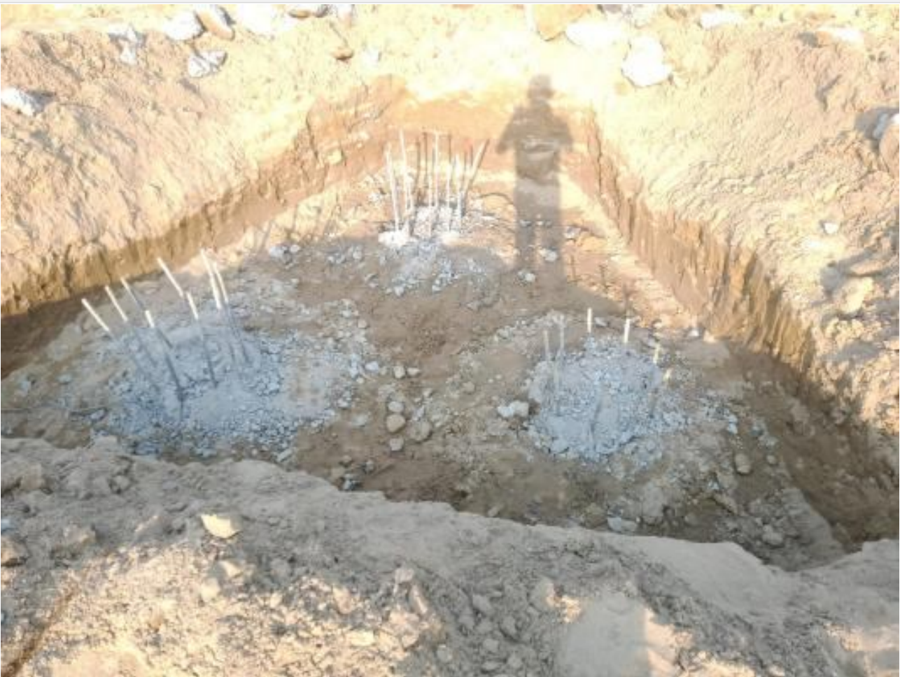
Dorm. Bldg. Pile head breaking on 07-05-23
