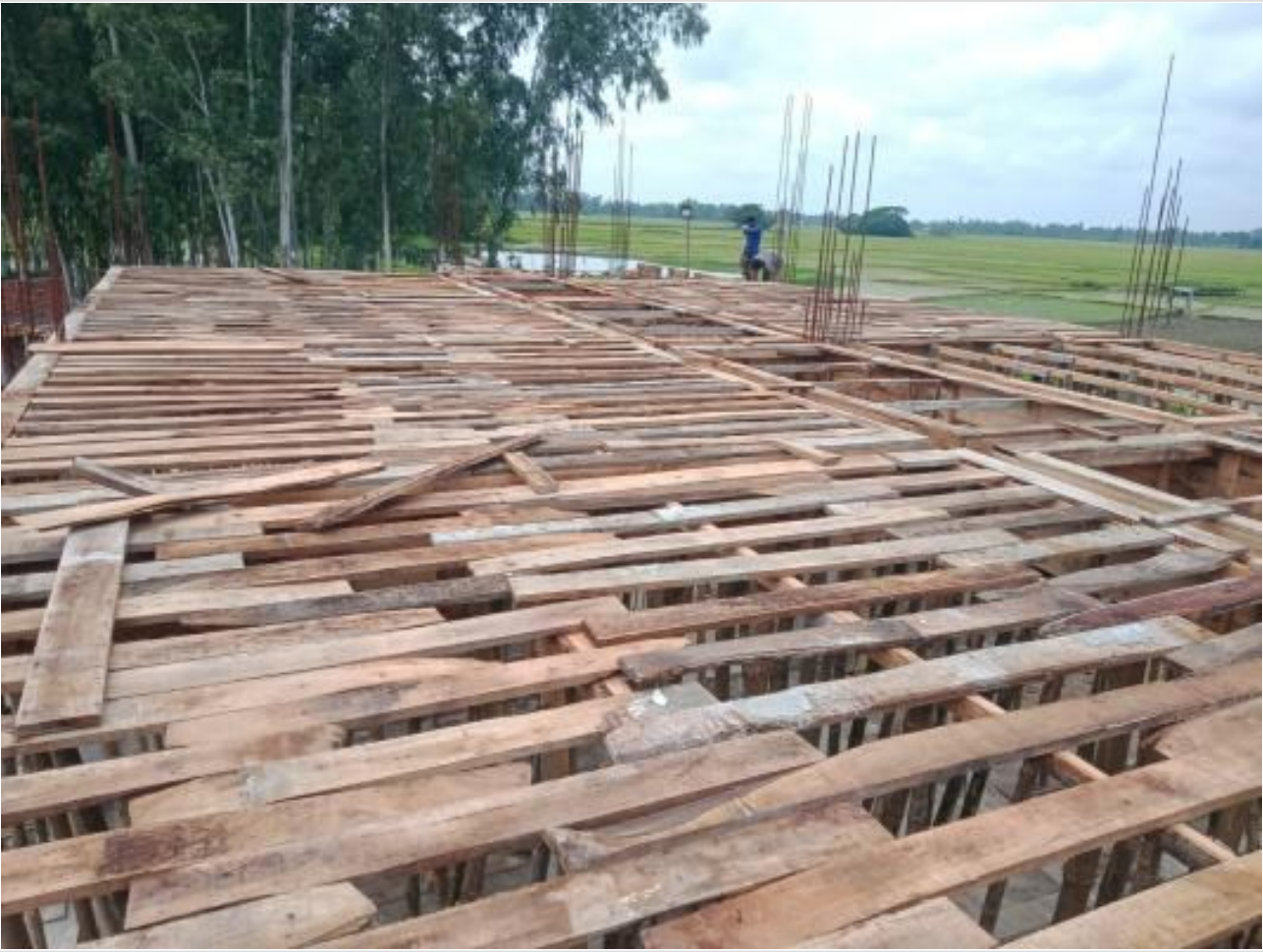
Dorm. Bldg shuttering work on 28-07-23
