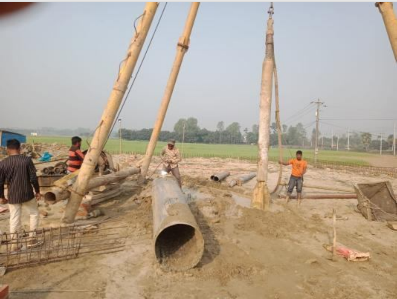
Pile boring work-CB(5+2) out of 69 nos p on 15-02-23
