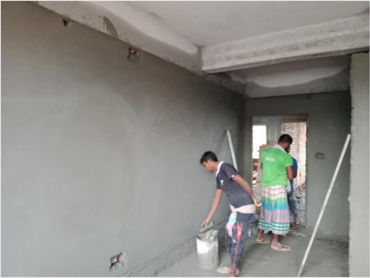
Comp. Bldg 1st fplaster work on 21-09-23
