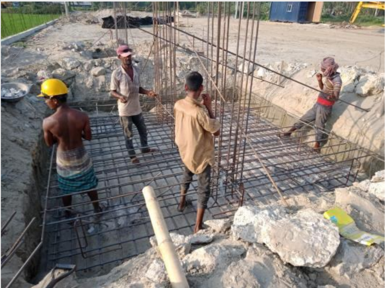
Pile cap rebar work on 14-04-23
