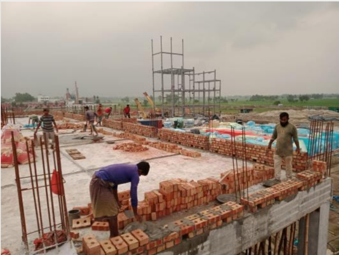
Comp-Parapet Brick-work on 14-08-23
