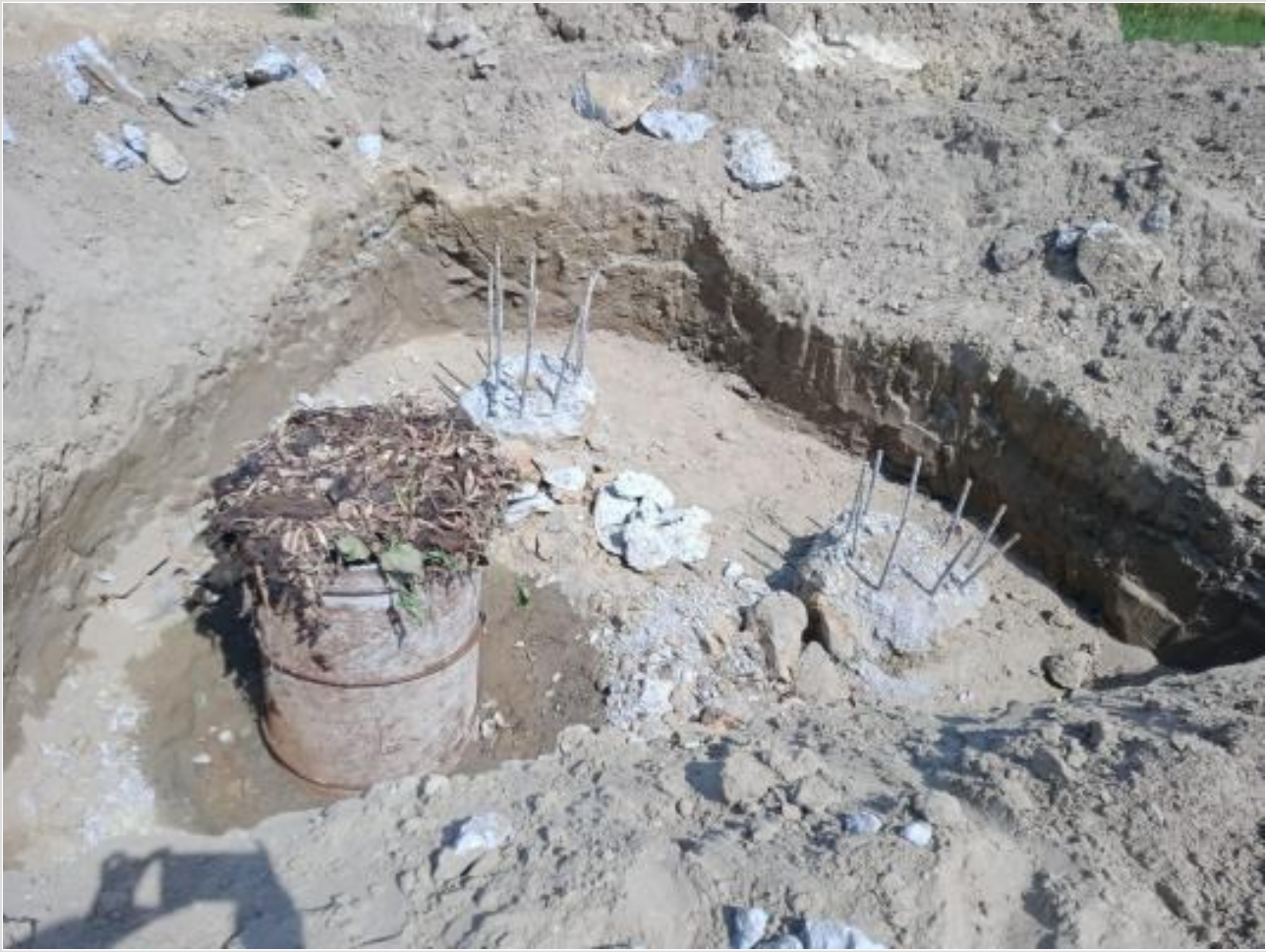
Pile head breaking on 10-05-23
