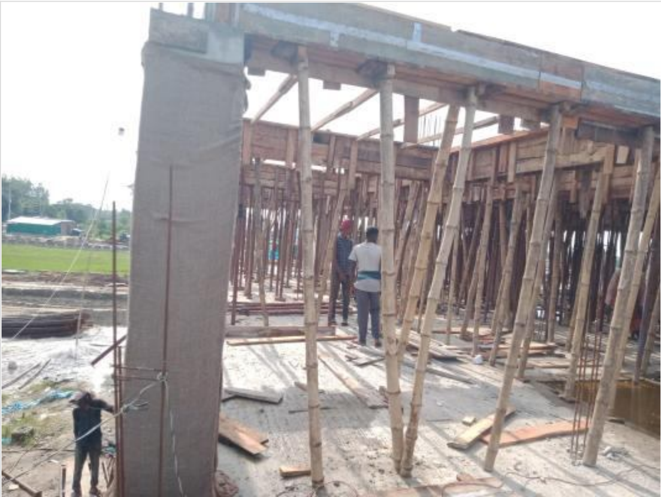
Comp. Bldg. 2nd floor slab shuttering wo on 19-07-23
