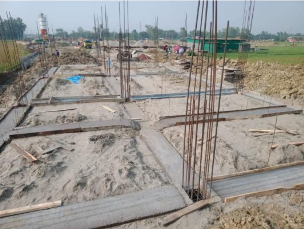
Dorm. Bldg. GB Bottom CC work on 03-06-23
