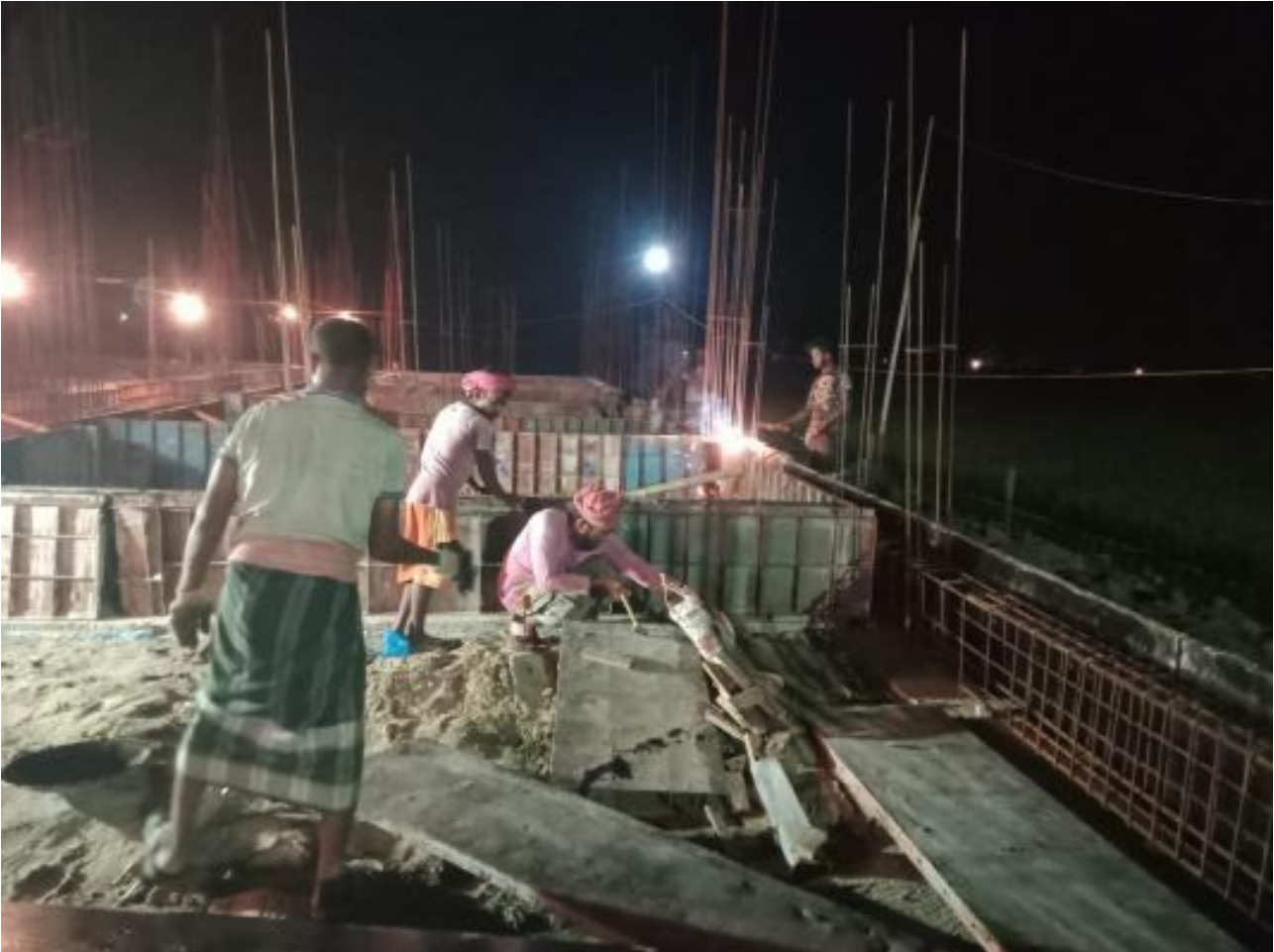
Com. GB Shuttering on 13-05-23
