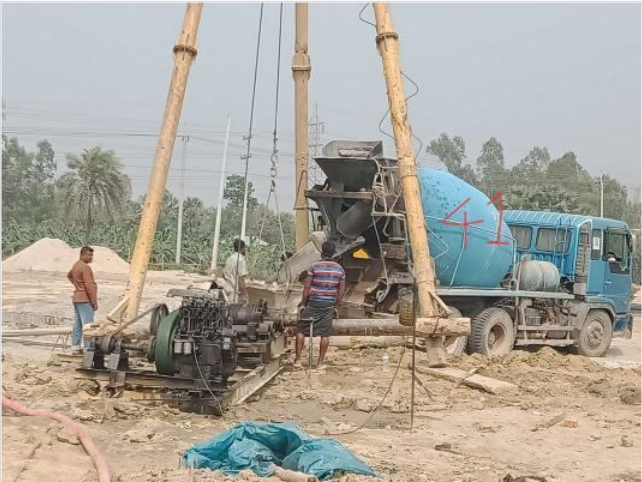
Ready mix concreting of pile on 03-03-23
