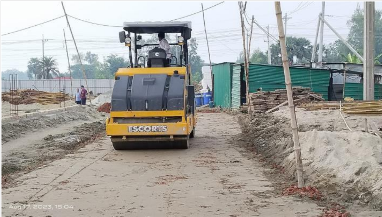
Sub-base Compaction on 17-08-23
