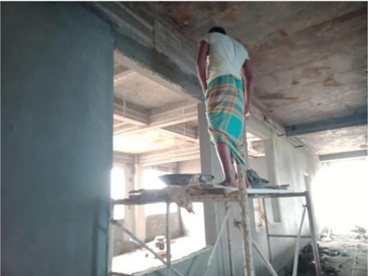
Comp. Bldg FF plastr wok on 19-09-23
