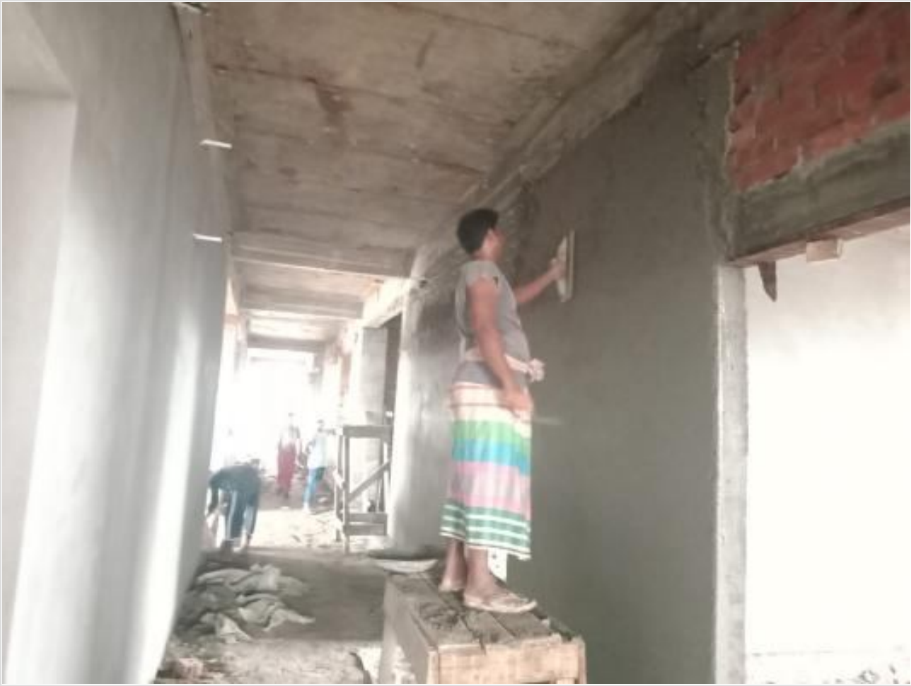
Comp. Bldg plaster work on 26-08-23
