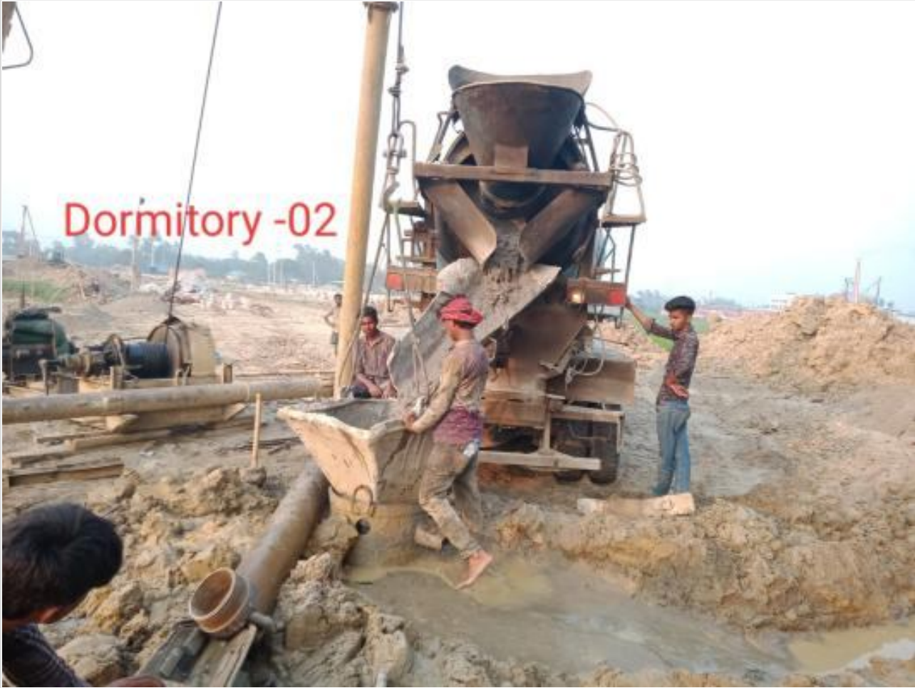
Ready mix concreting of pile on 25-03-23
