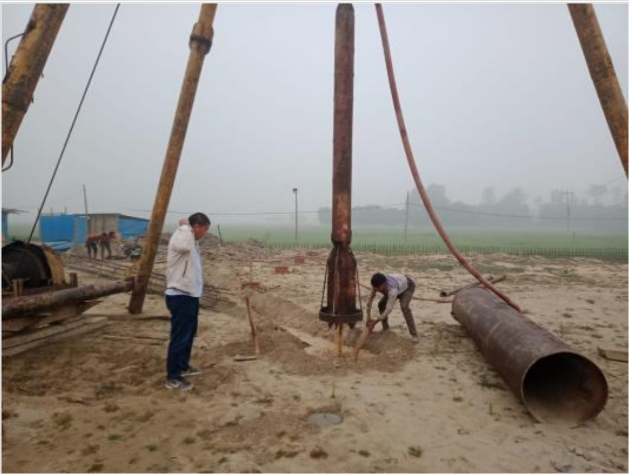
Pile Driving Starting on 09-02-23
