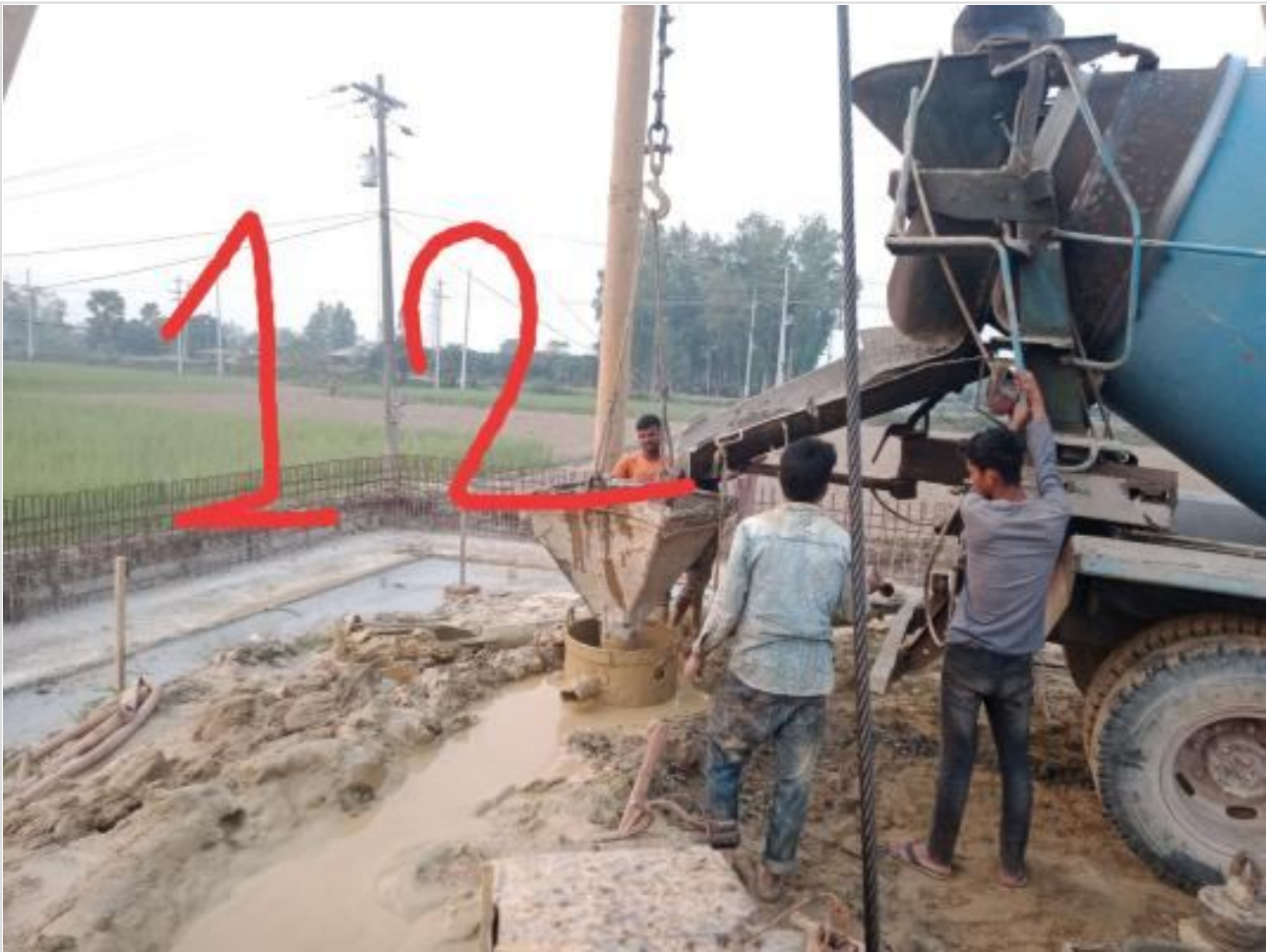
Ready mix concreting of pile on 17-02-23
