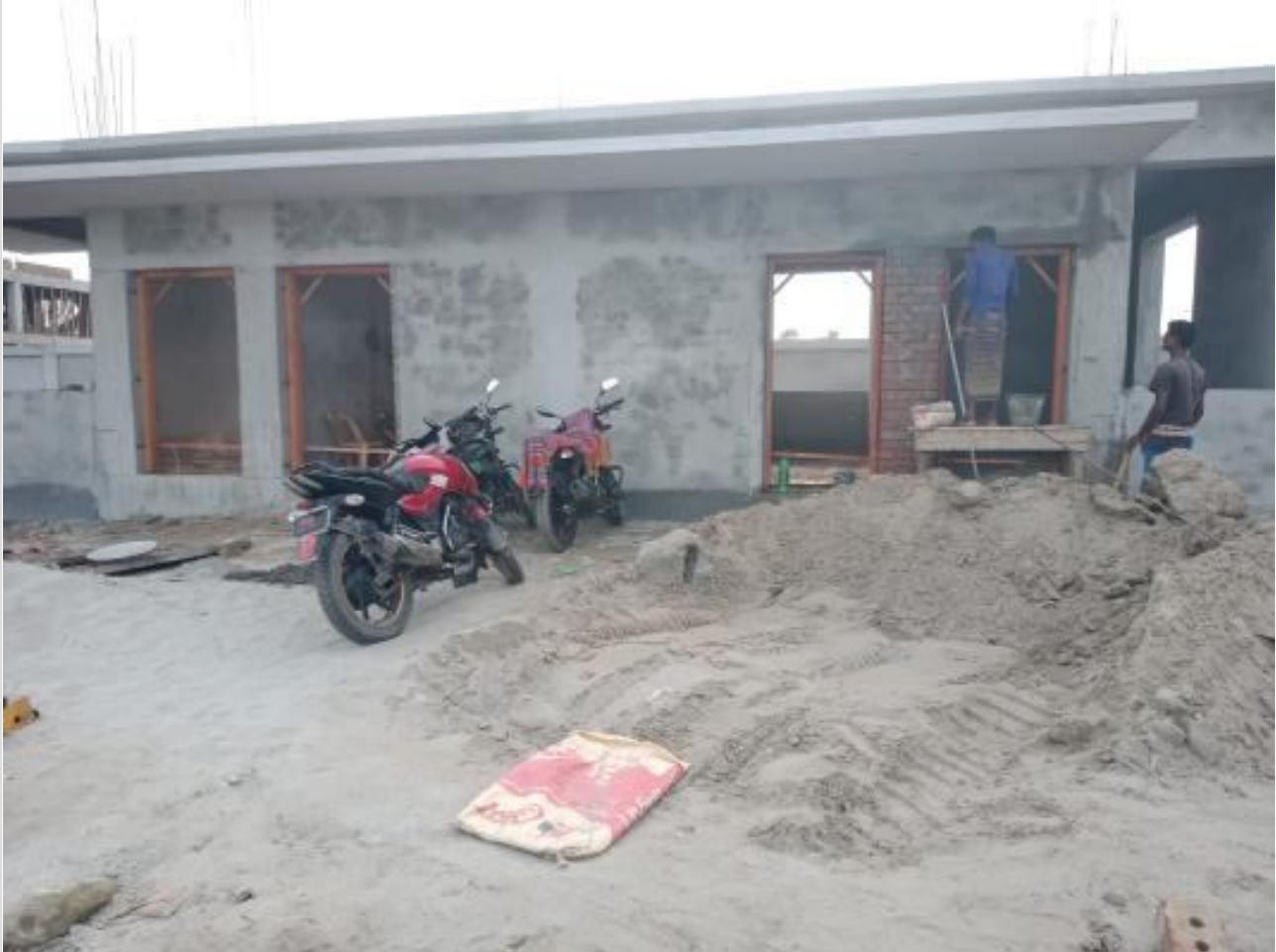
Gate House-Door Frame Fixing on 20-08-23
