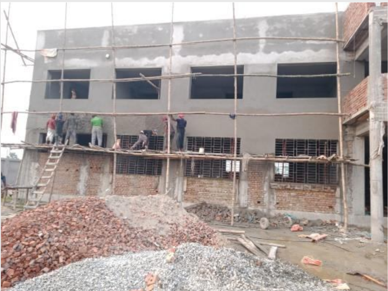
Comp. Bldg. Outside plaster work on 16-10-23
