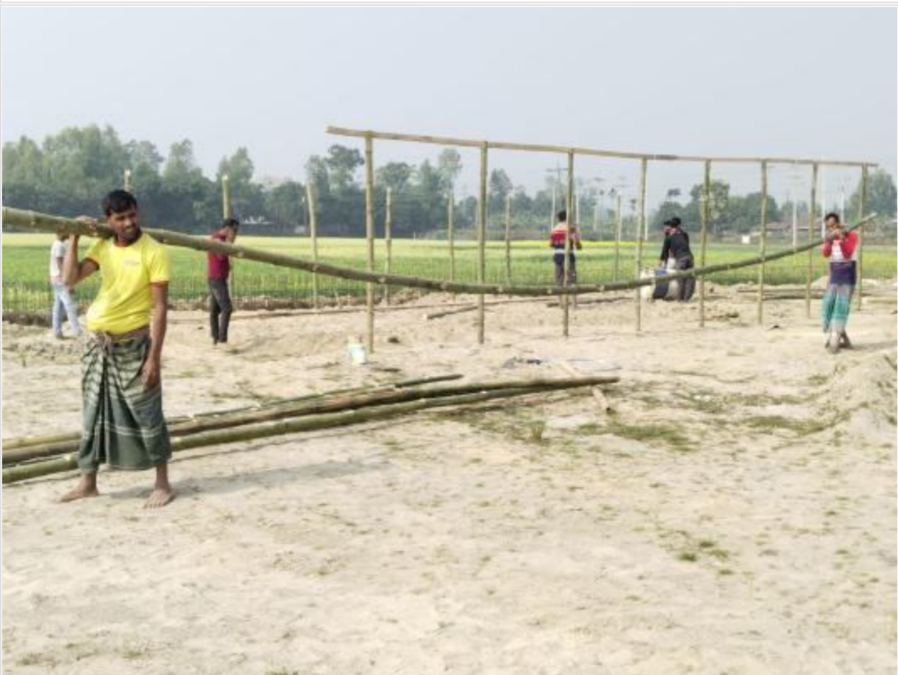
Shed making on 17-01-23
