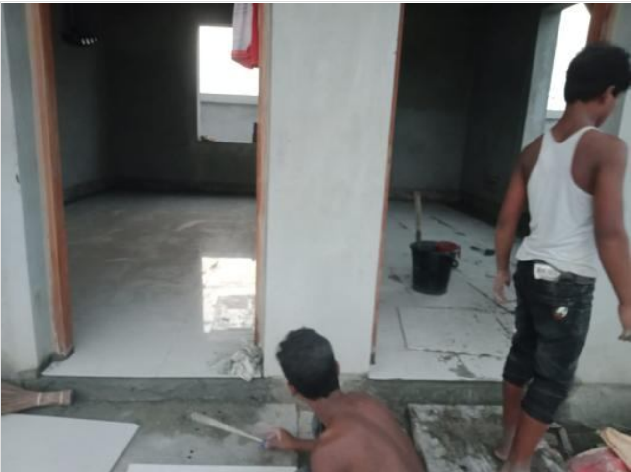
Gats house files work on 26-09-23
