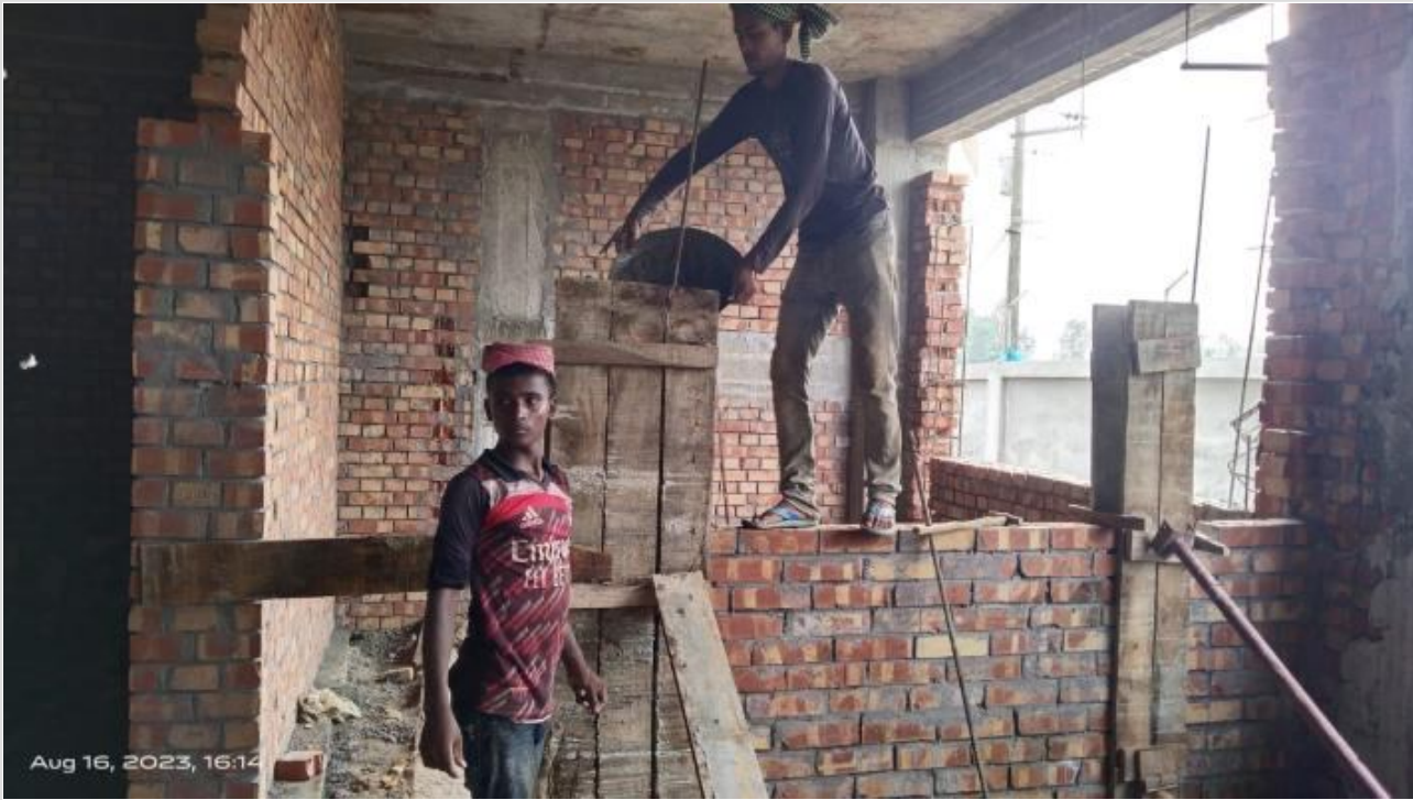
Comp-GF Column Concreting on 16-08-23
