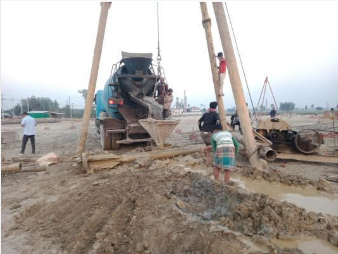
Ready mix concreting of pile on 14-02-23
