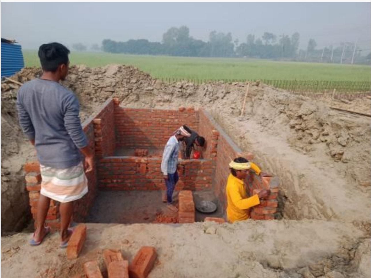
Mud Tank making on 06-02-23
