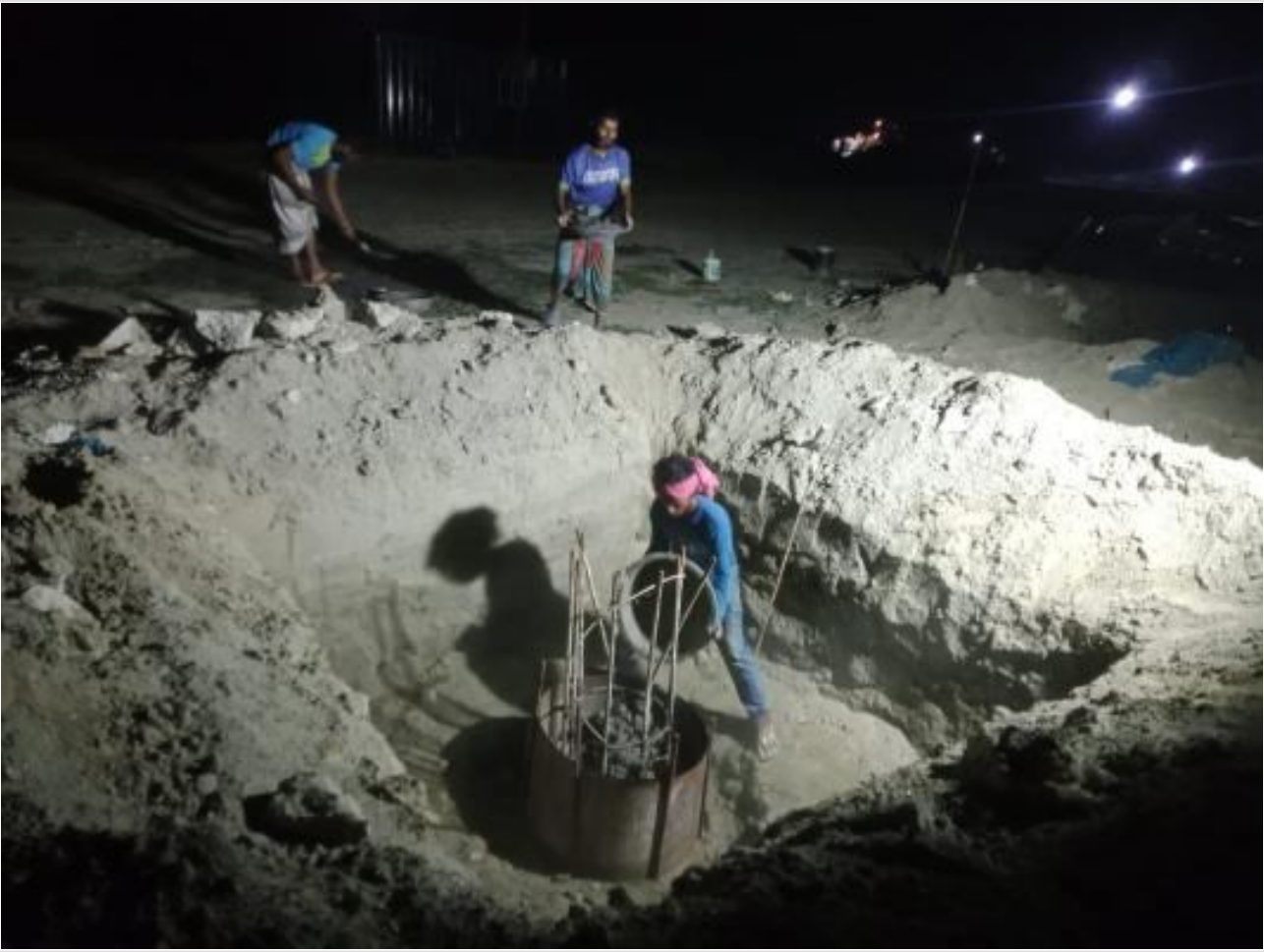
Gate pile Cap cc work on 08-05-23
