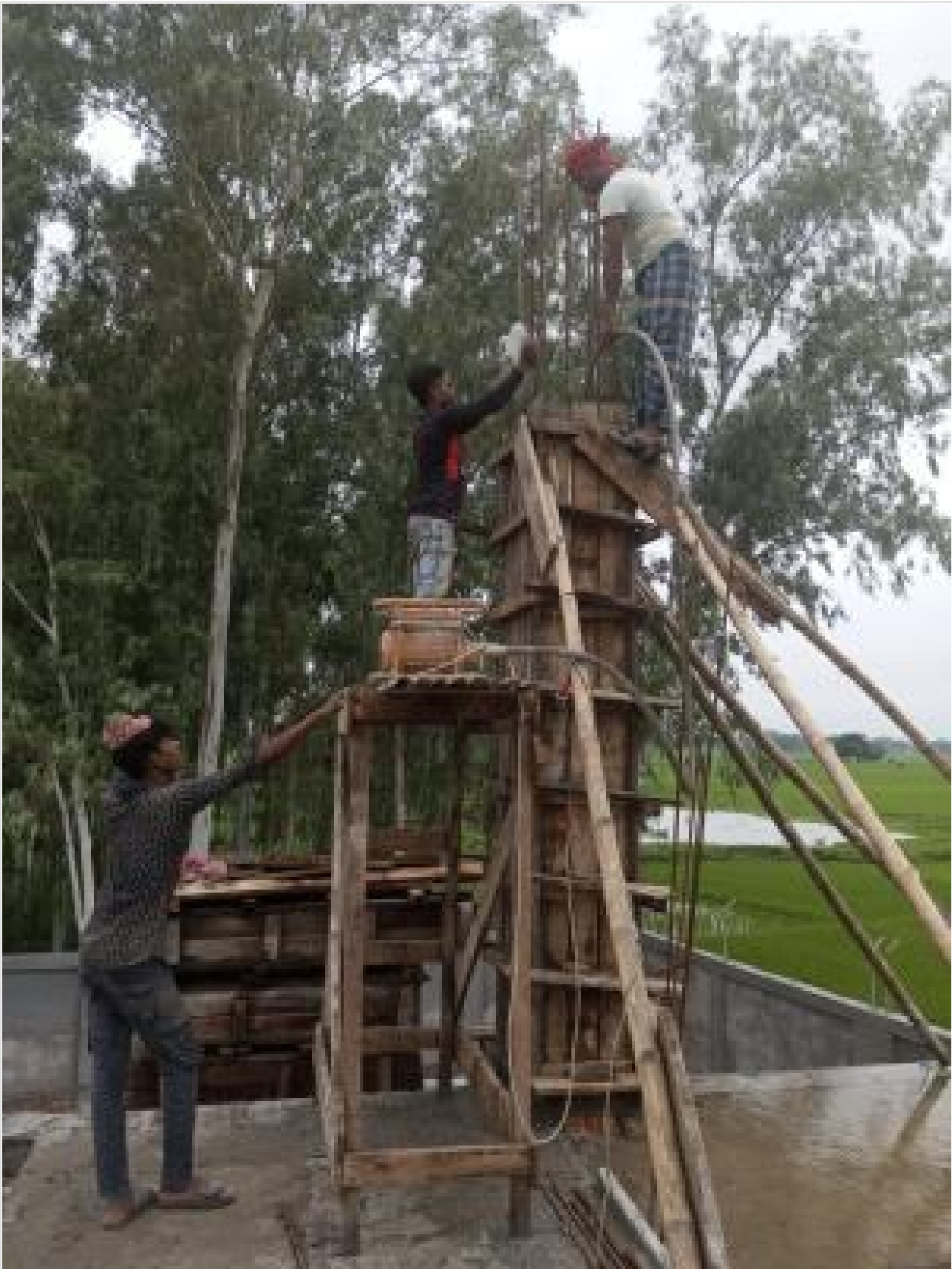
Column casting work on 25-08-23
