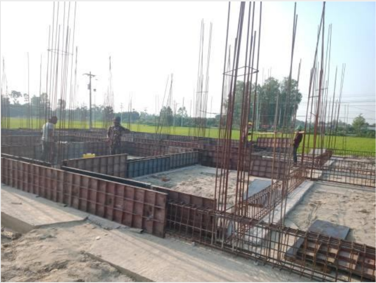
Comp. GB Shuttering on 07-05-23
