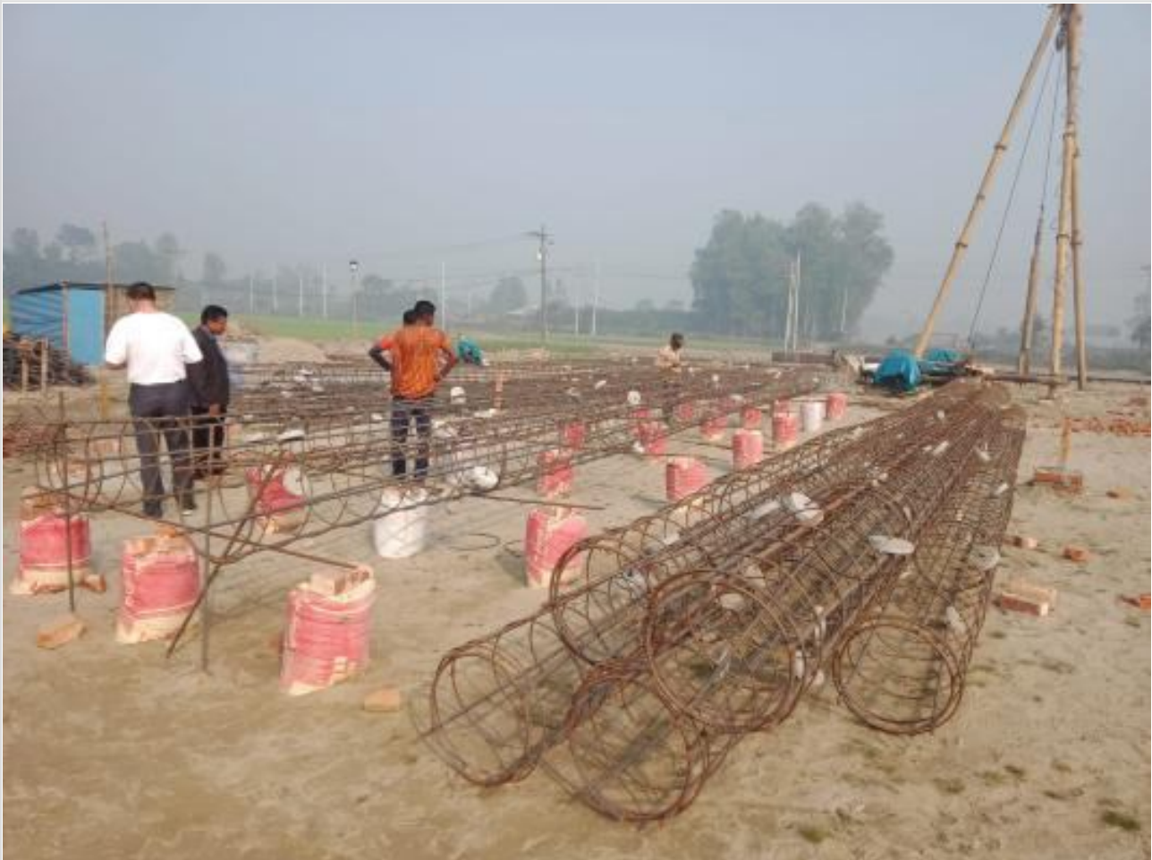
Pile Re-bar Work on 12-02-23
