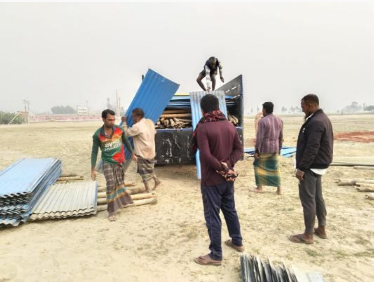
Unloading Materials on 14-01-23
