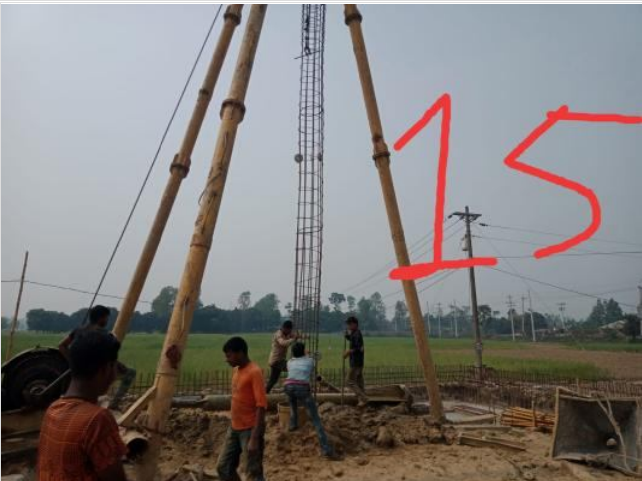
Com. Bldg. 15th pile boring on 19-02-23
