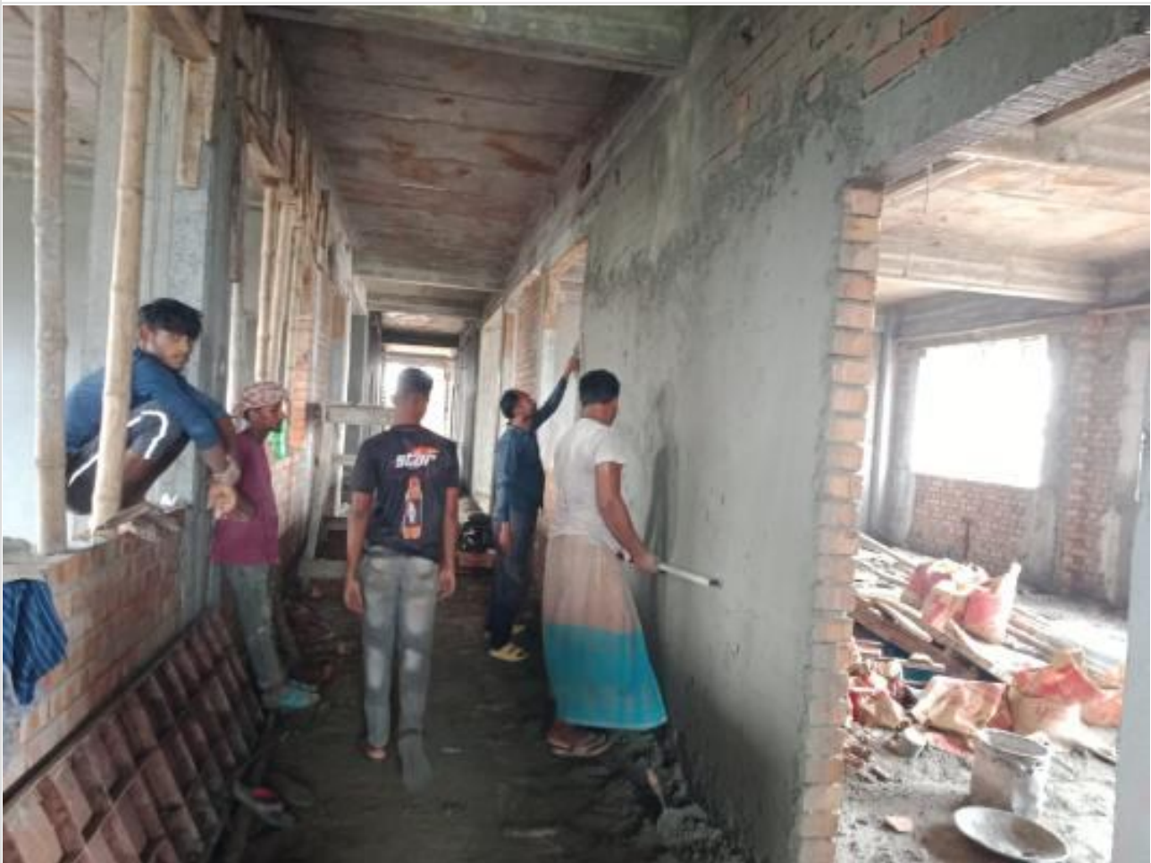
Comp. Bldg. GF plaster work on 27-08-23
