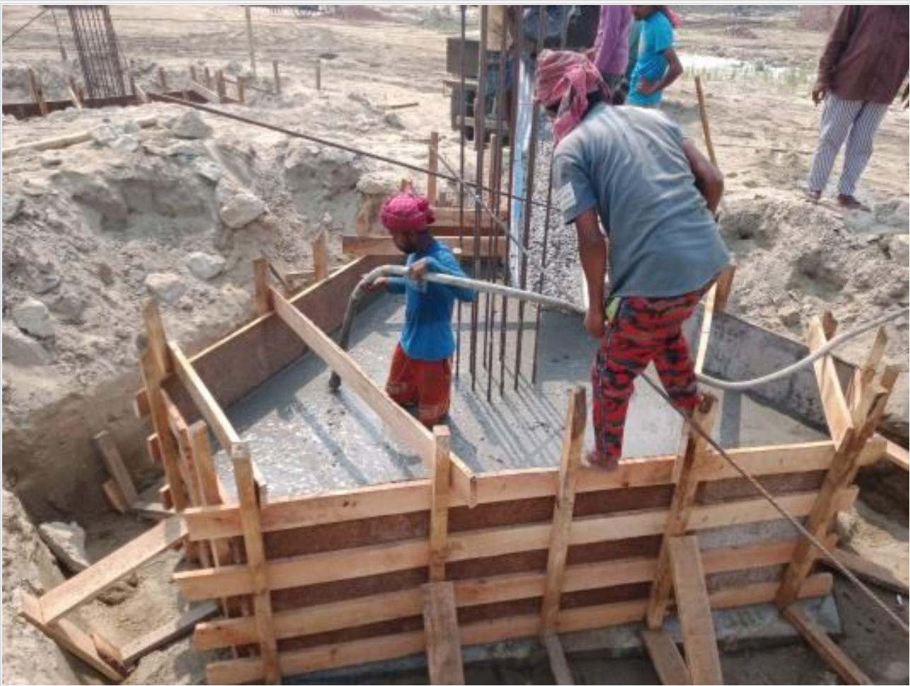
Comp. Bldg. Pile cap casting on 16-04-23
