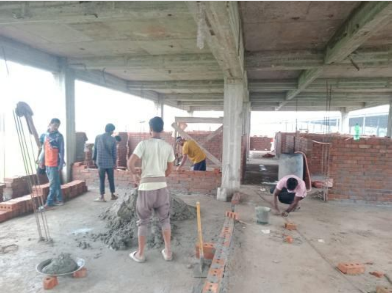
Dorm. 1st floor brick work on 07-10-23
