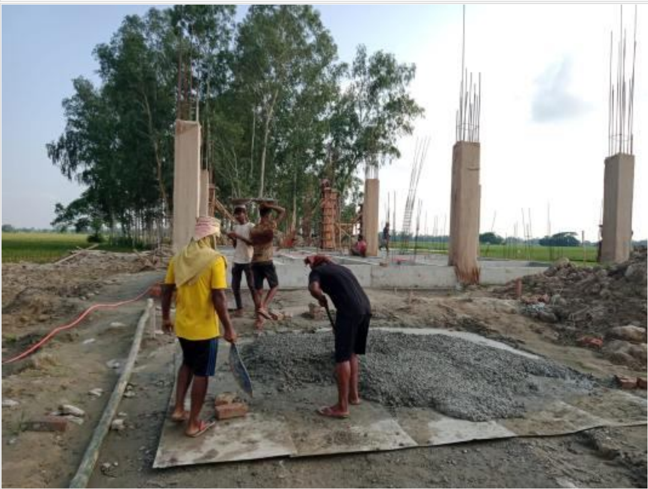
Dorm. Bldg. Column Casting on 23-06-23
