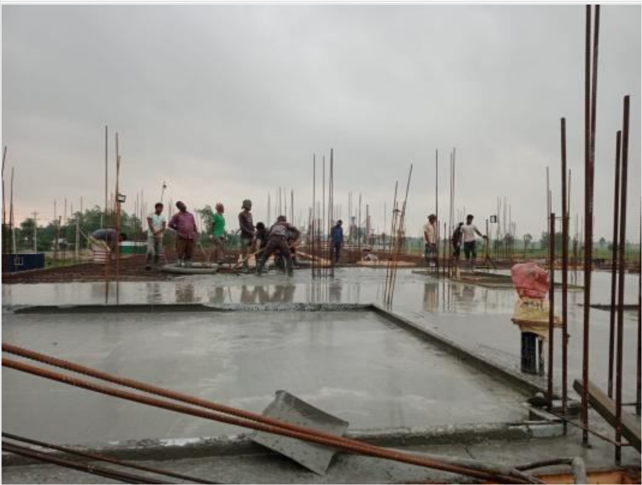
Com. Bldg. 1st floor slab casting on 27-06-23
