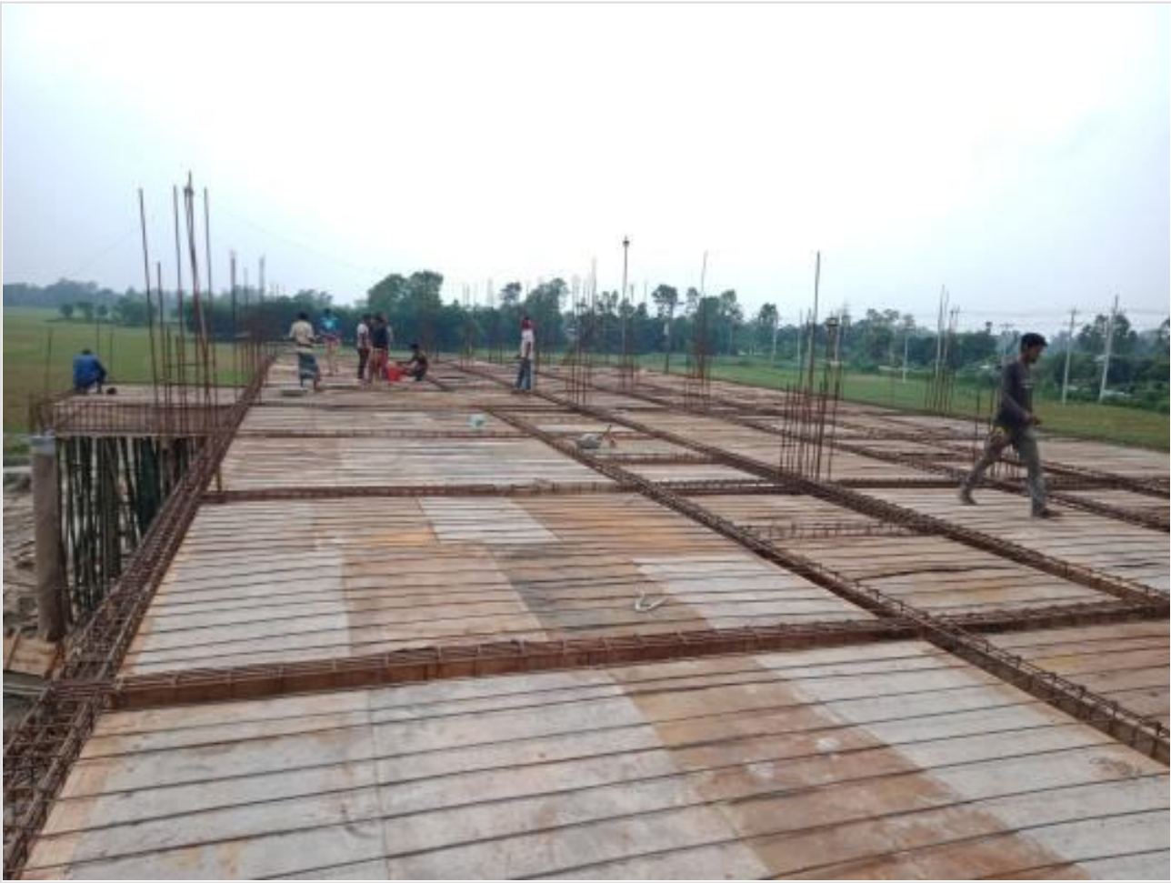
Comp. Bldg. Slab beam shuttering on 15-06-23
