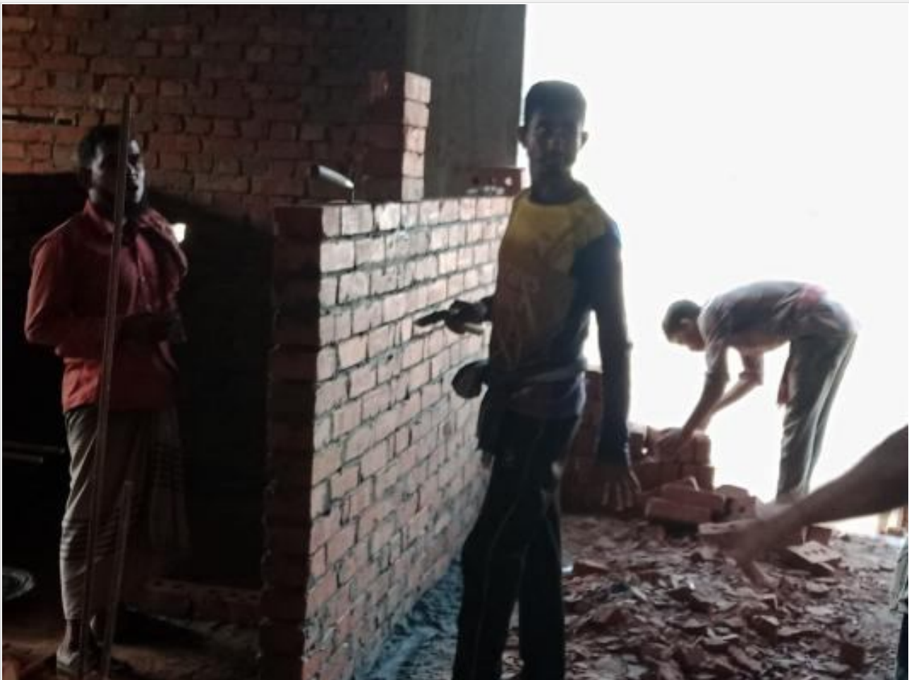
Dorm. Bldg. 1st floor brick work on 13-09-23
