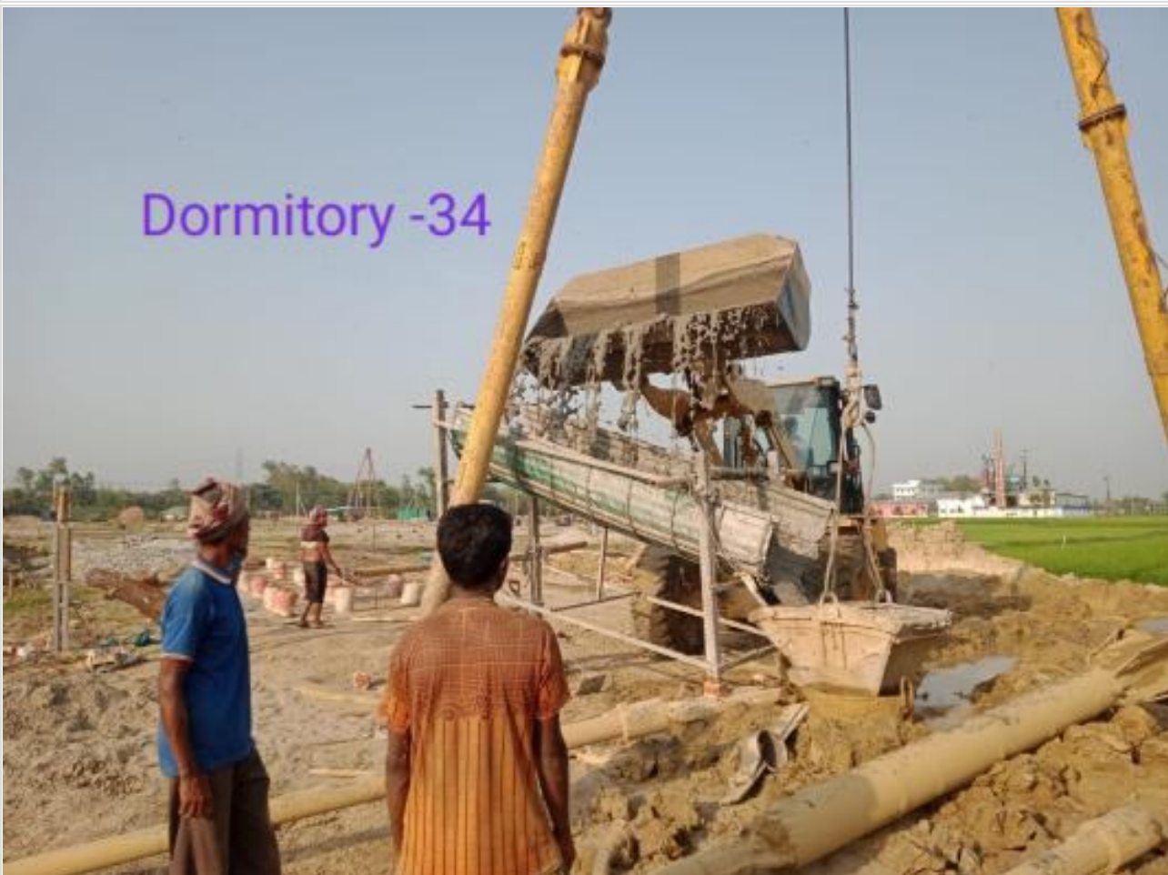
Dorm. Bldg. 32nd pile concreting on 09-04-23
