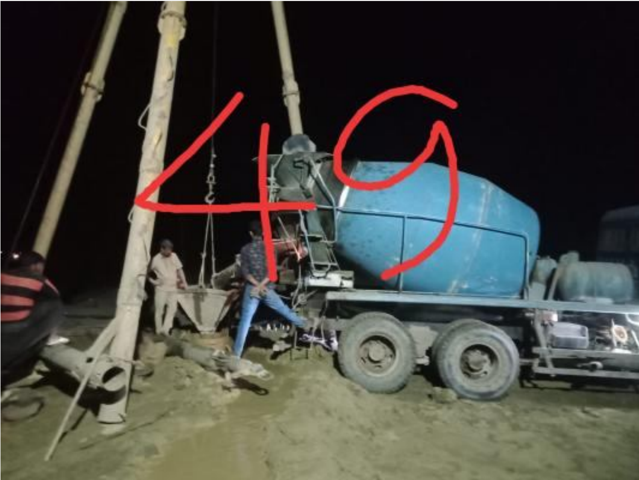
Ready mix concreting of pile on 08-03-23
