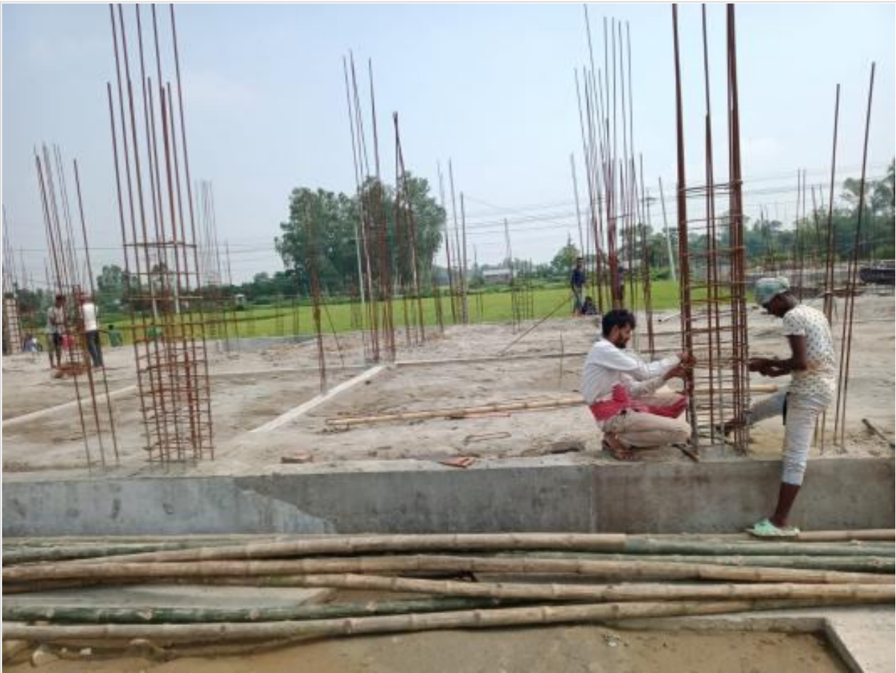
Comp. Bldg column work on 25-05-23
