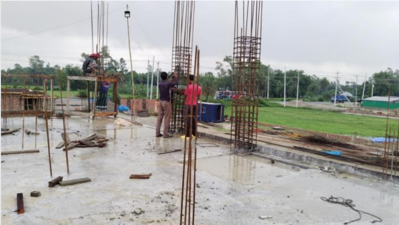
Comp Bldg-1st floor Column Re-bar work on 06-07-23
