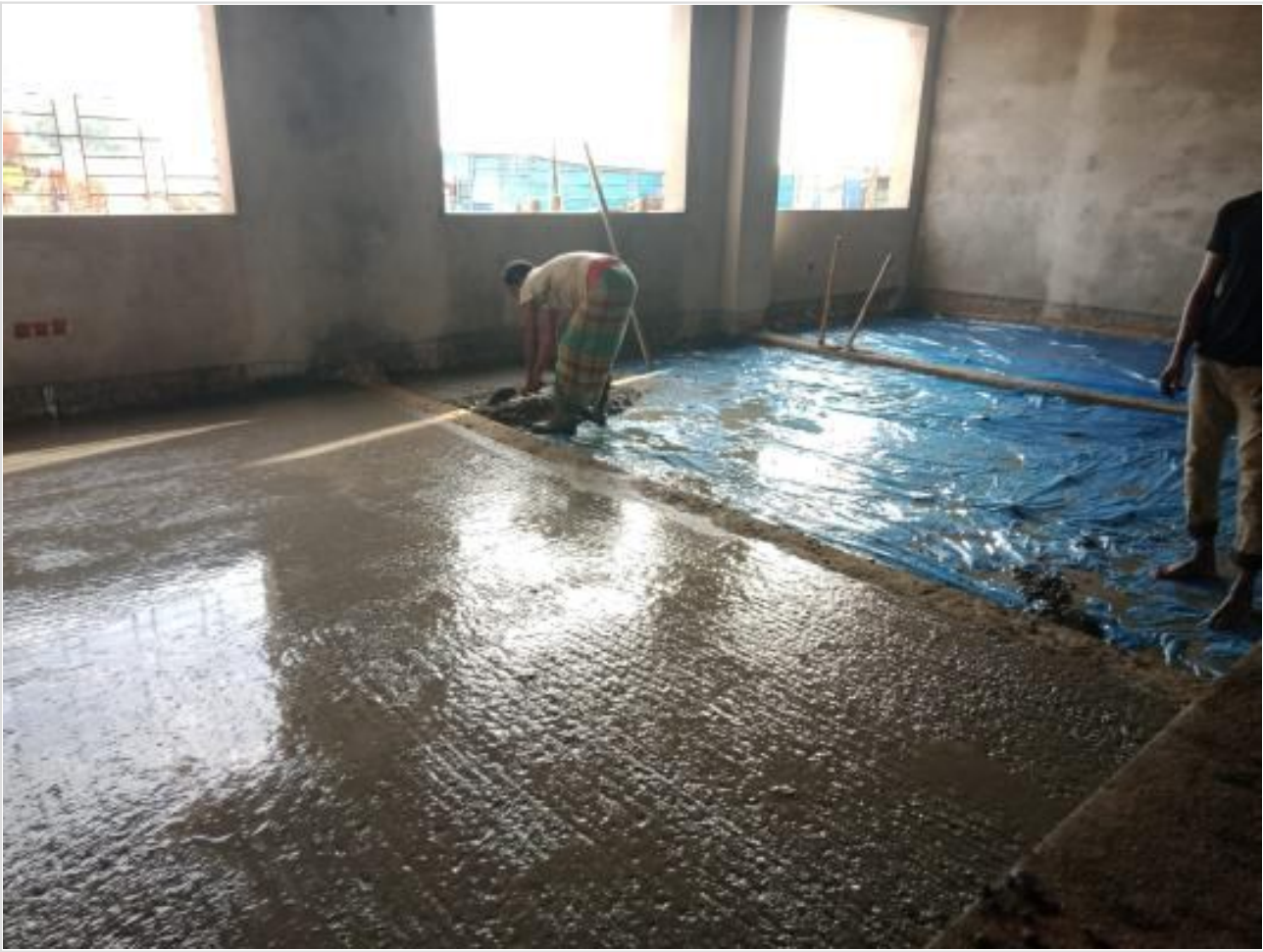
Comp. GF concreting on 29-09-23
