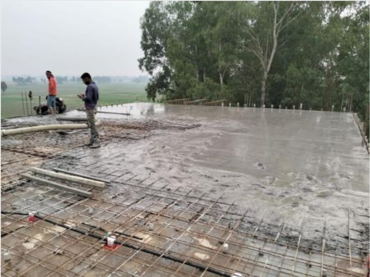
Dormitory-3rd Floor Slab Concreting on 23-12-23
