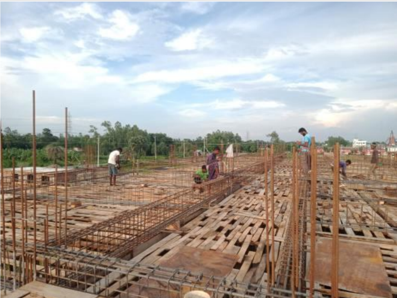
Comp. Bldg. 2nd Floor rebar work on 28-07-23
