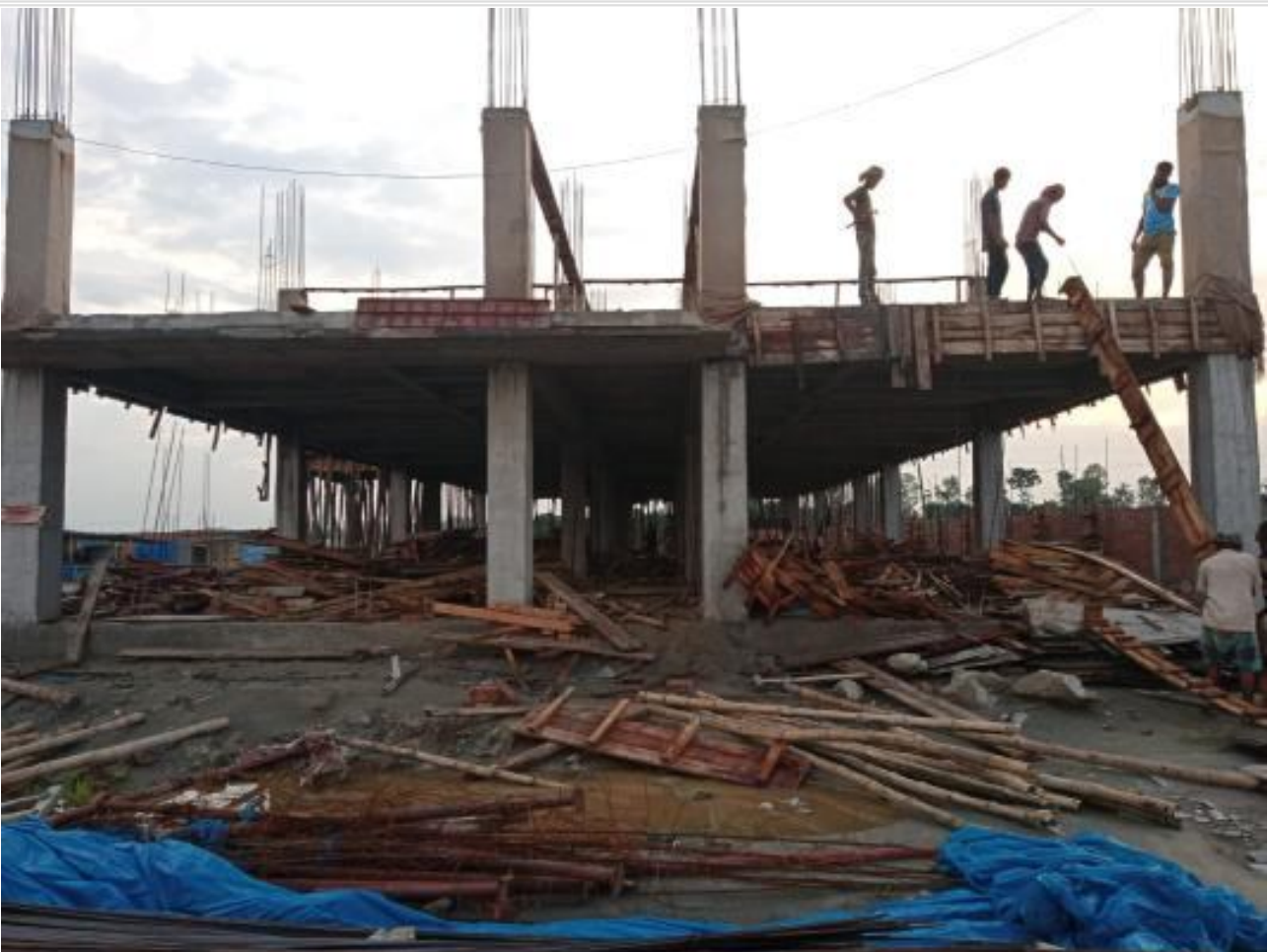
Comp. Bldg. 1st floor column work on 14-07-23
