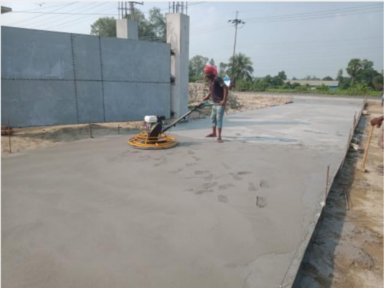
Road casting work on 18-10-23
