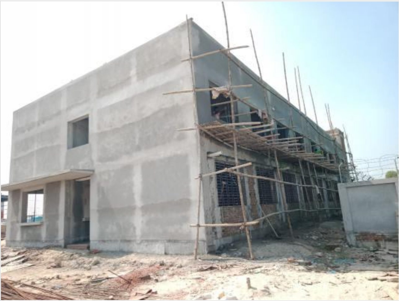
Comp. Building-Outside Plastering on 20-10-23
