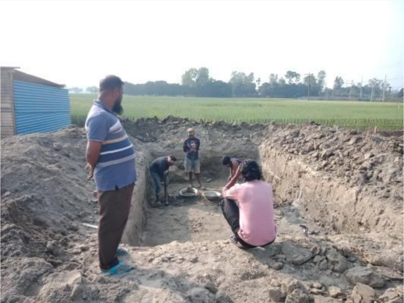
Excavation for Pile Mud Tank on 03-02-23
