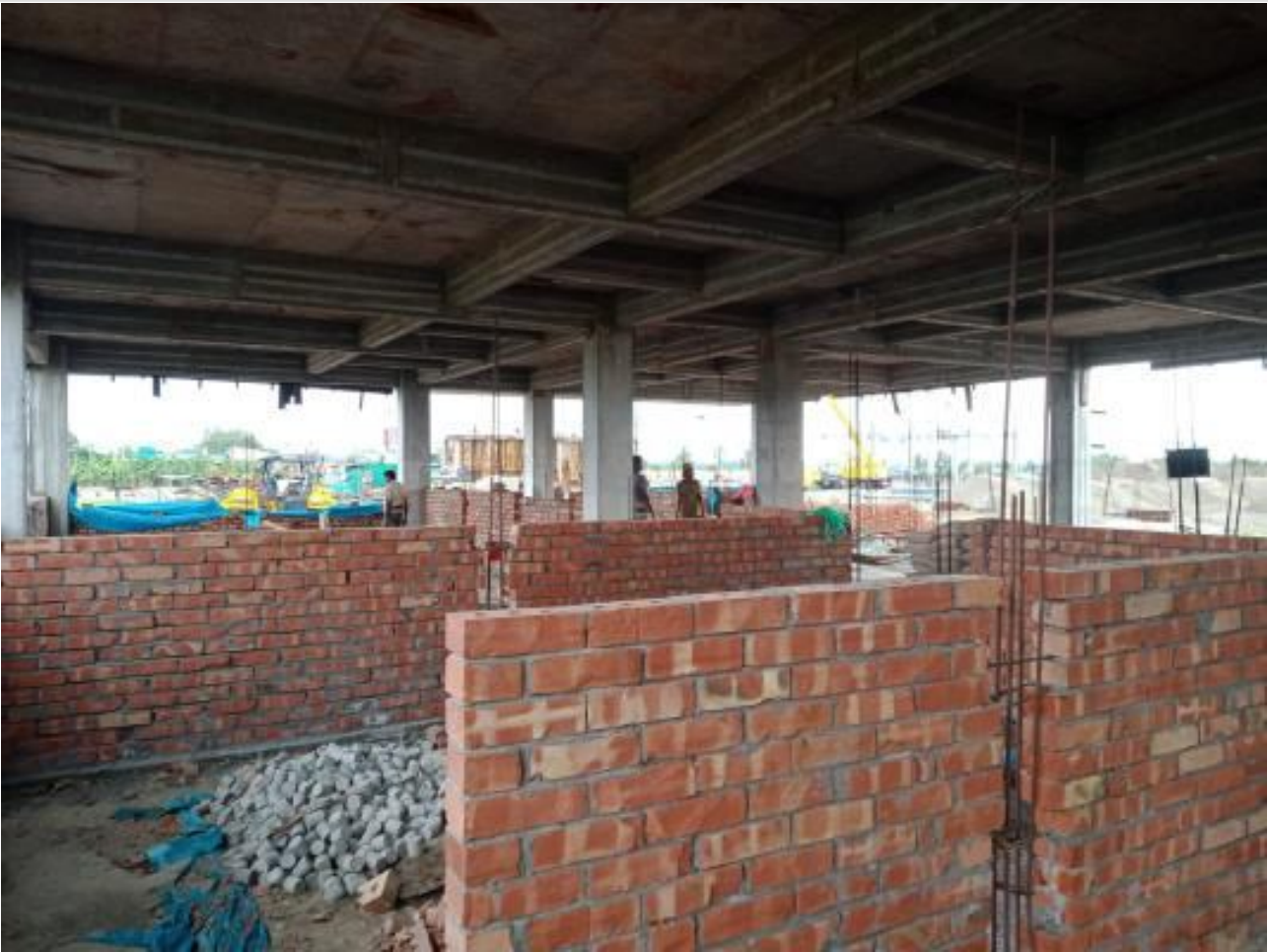
Comp. Bldg. GF Brick work on 21-07-23
