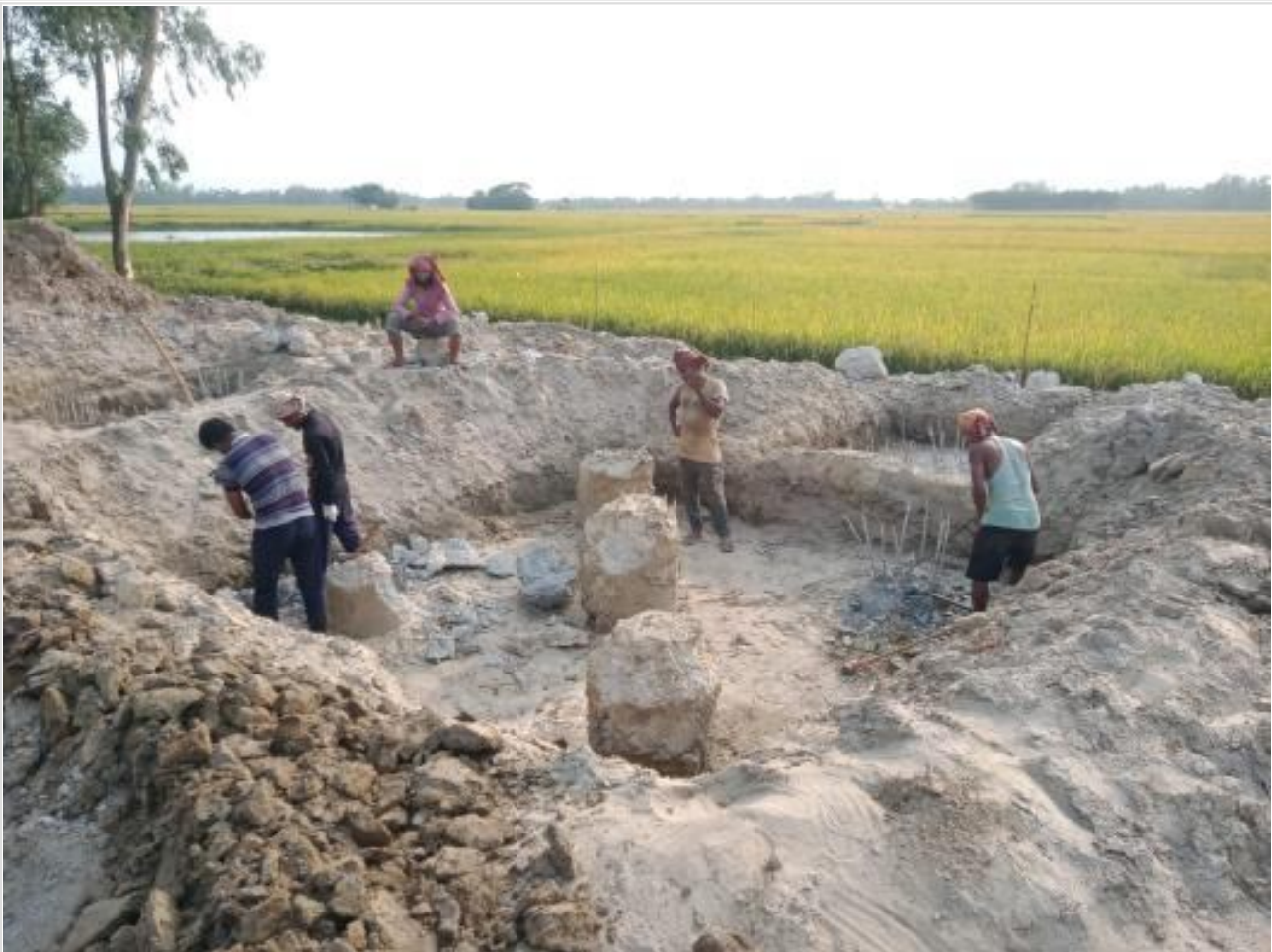
Dorm Bldg pile head breaking on 15-05-23
