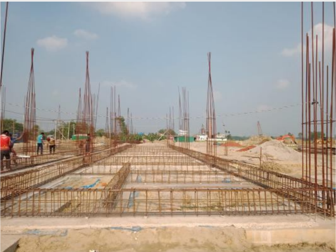
Comp. Bldg. GB Re-bar work on 05-05-23
