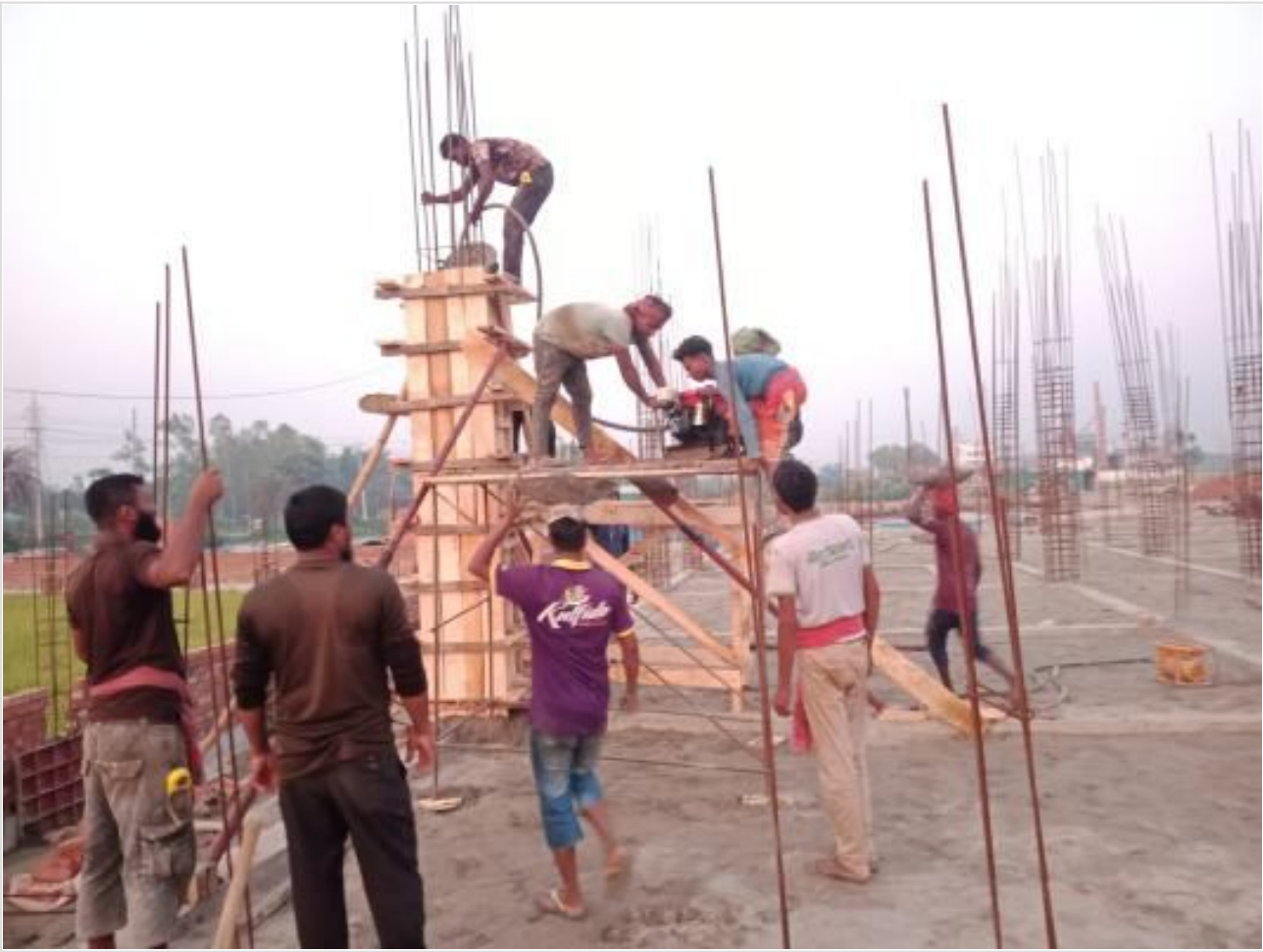
Comp. Bldg column casting on 28-05-23
