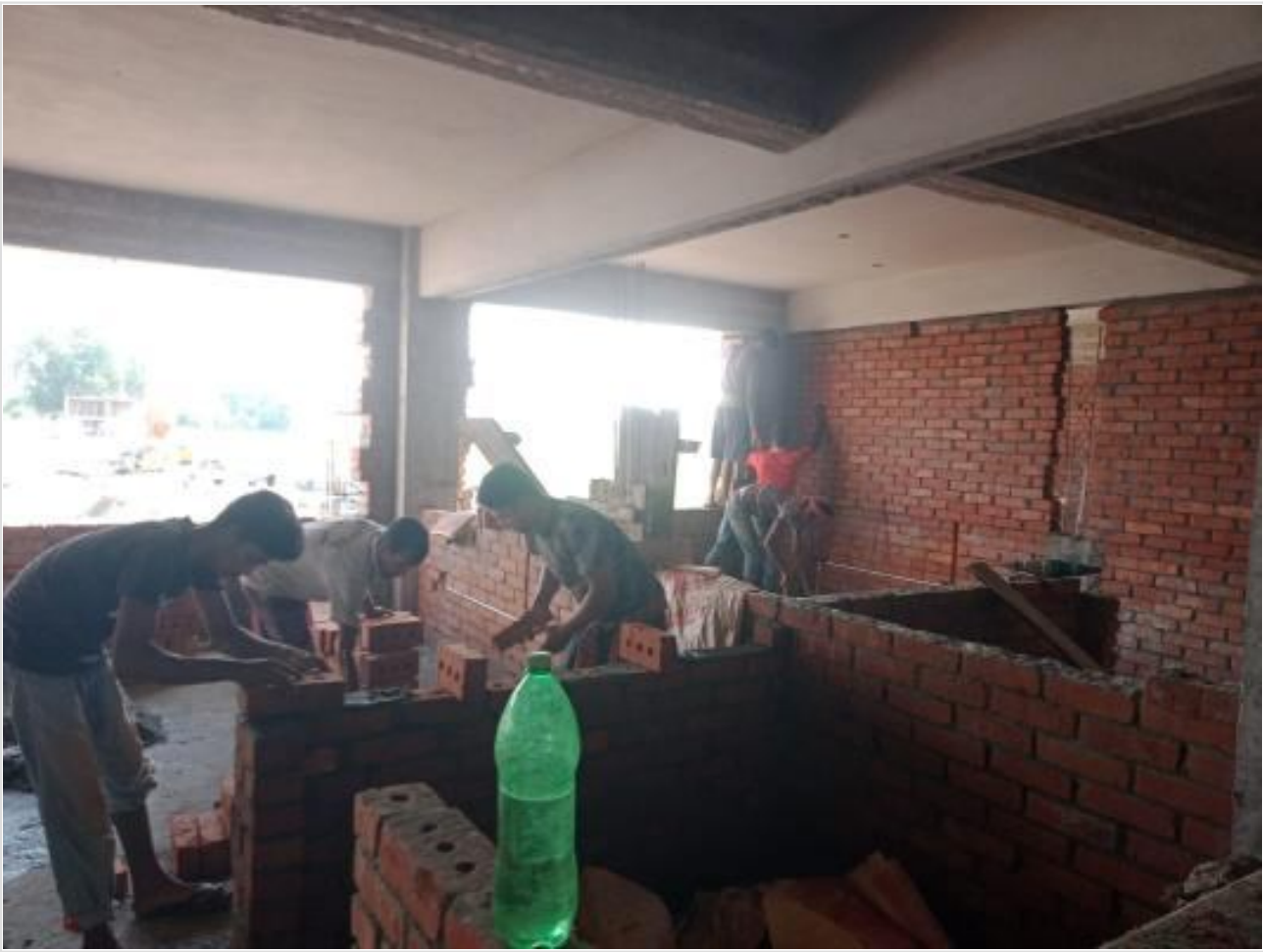
Comp. Bldg. FF Brick work on 09-09-23
