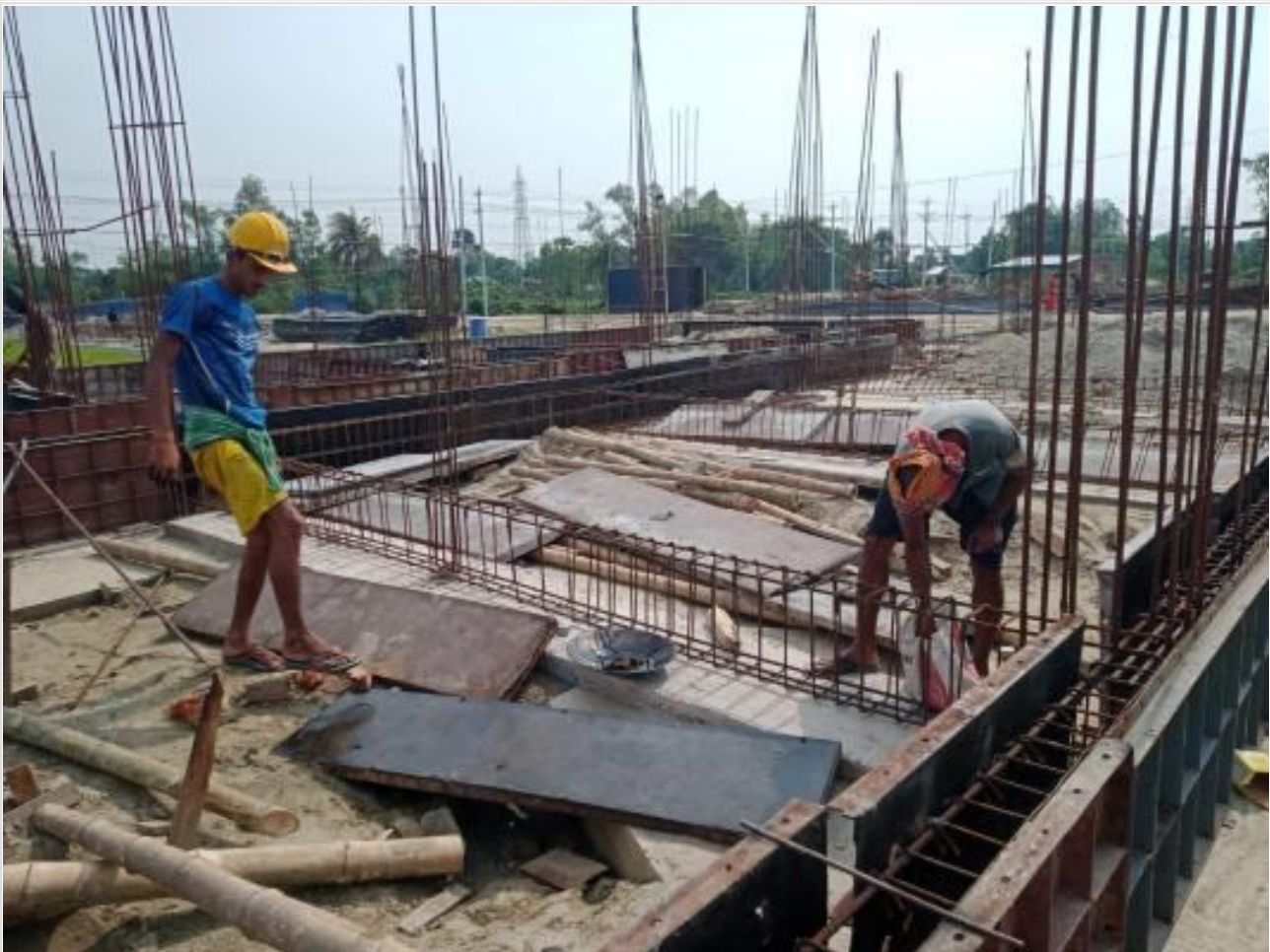
Comp. Bldg. GB Shuttering work on 14-05-23
