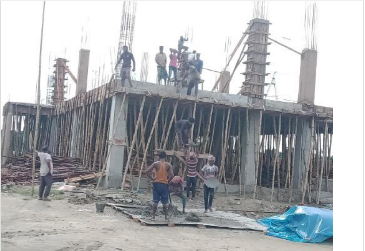
Comp. Bldg. 1st floor column casting on 12-07-23
