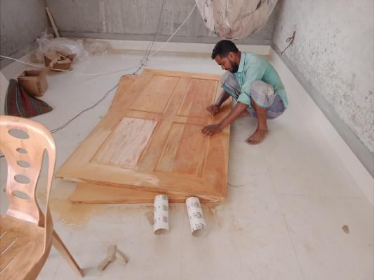
Comp. Bldg. Door shutter work on 26-10-23
