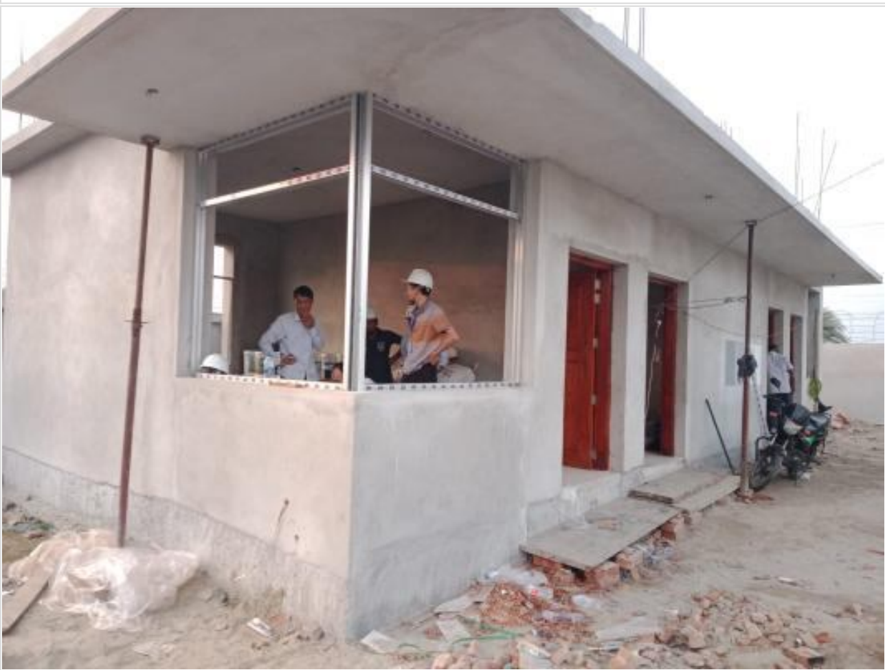
Gate House Thai work on 07-11-23
