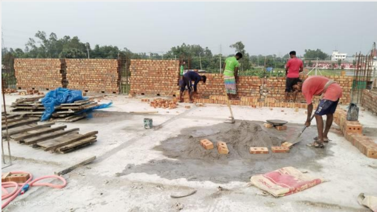
Comp-Parapet Brick-work on 17-08-23
