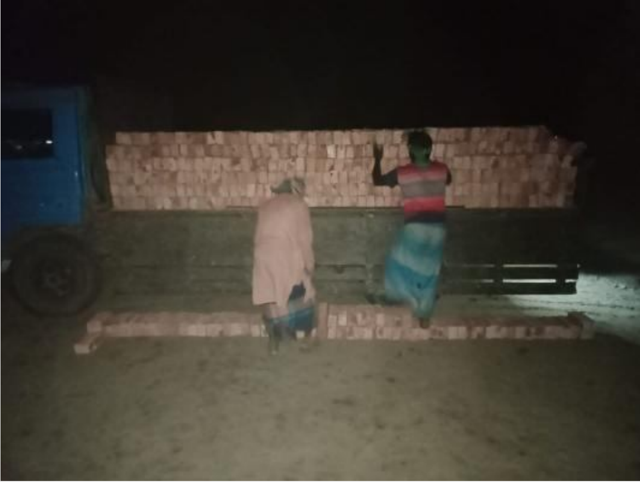
Brick un-loading on 09-01-23
