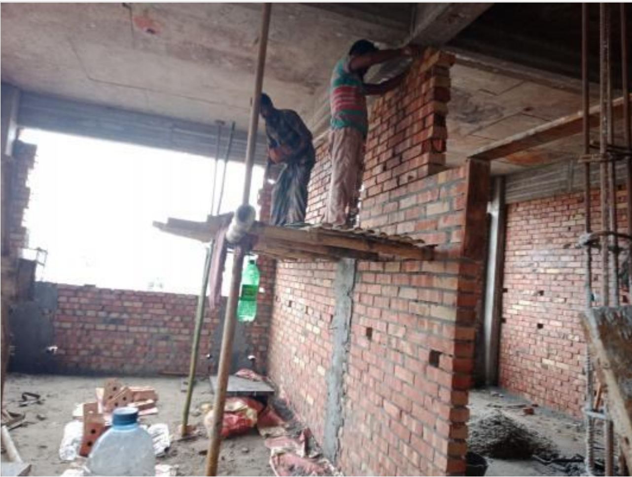
Comp-GF-Brick Work on 07-08-23
