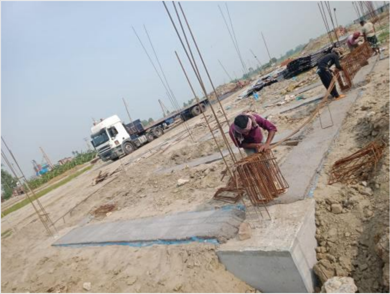
Re-bar work on 13-05-23
