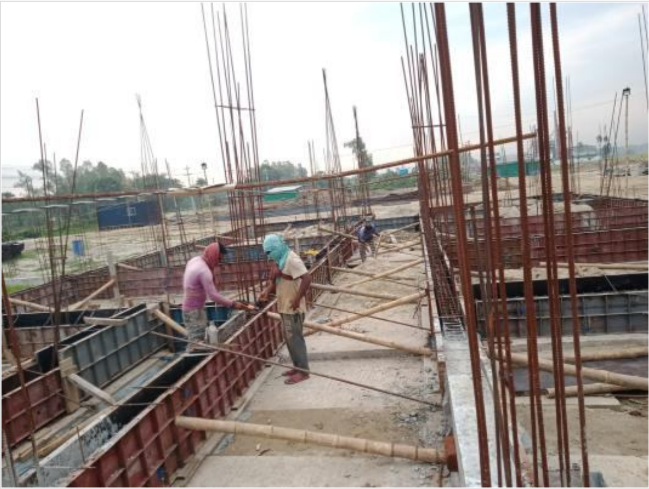
Com Bldg GB Shuttering on 15-05-23
