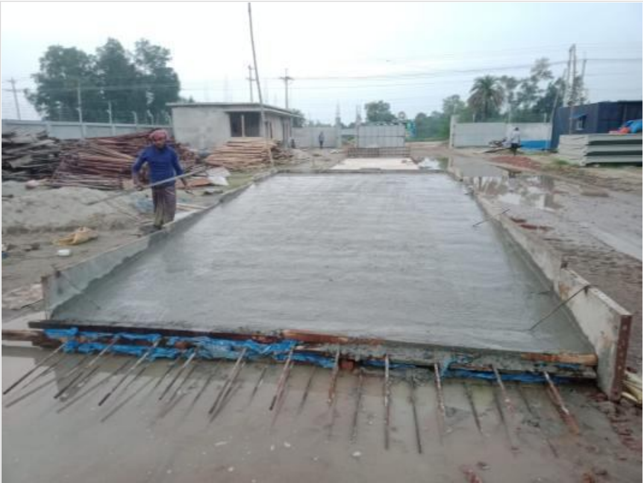
Weight scale concreting on 26-09-23
