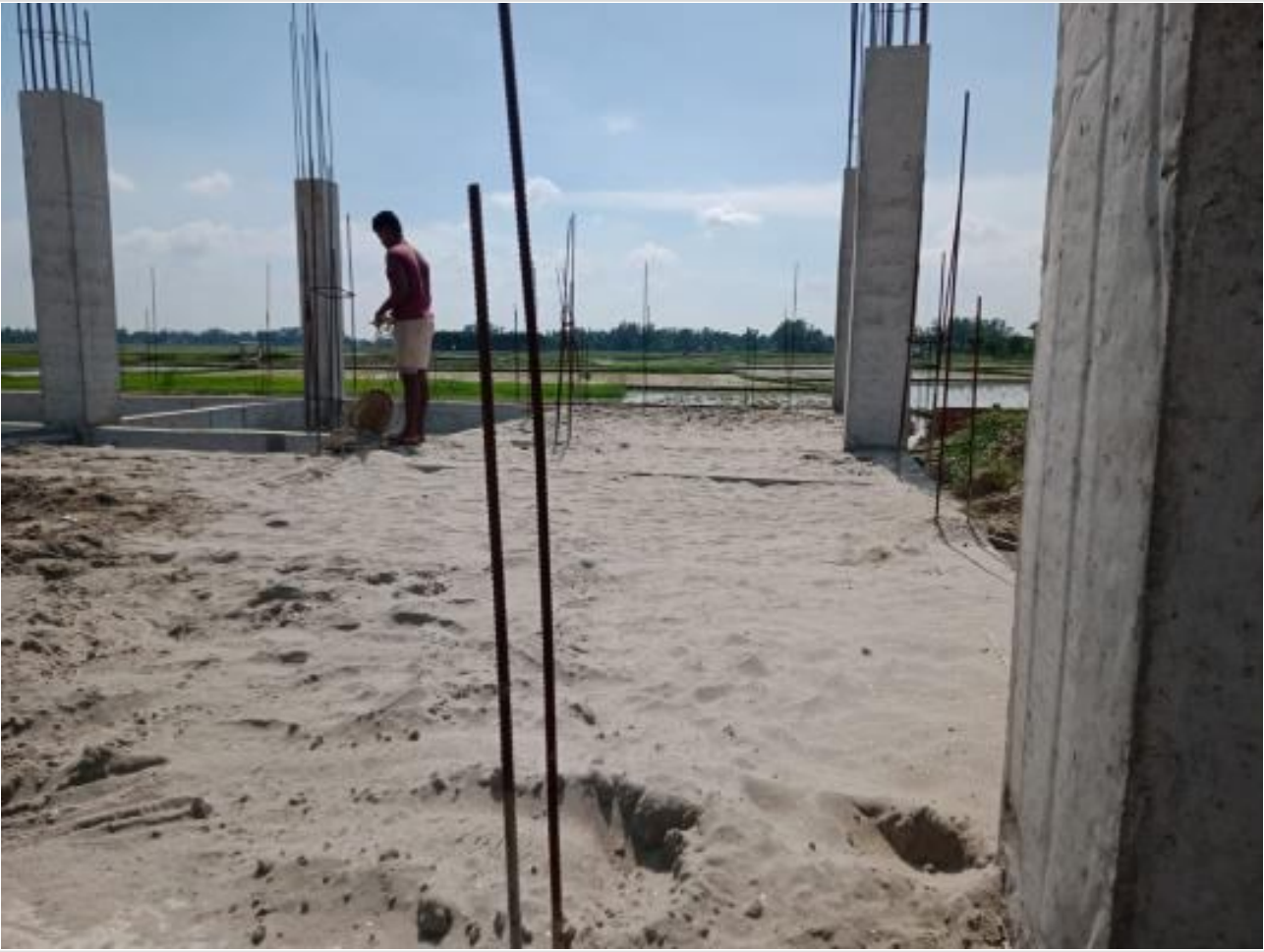
Dorm. Bldg. Sand filling on 18-07-23
