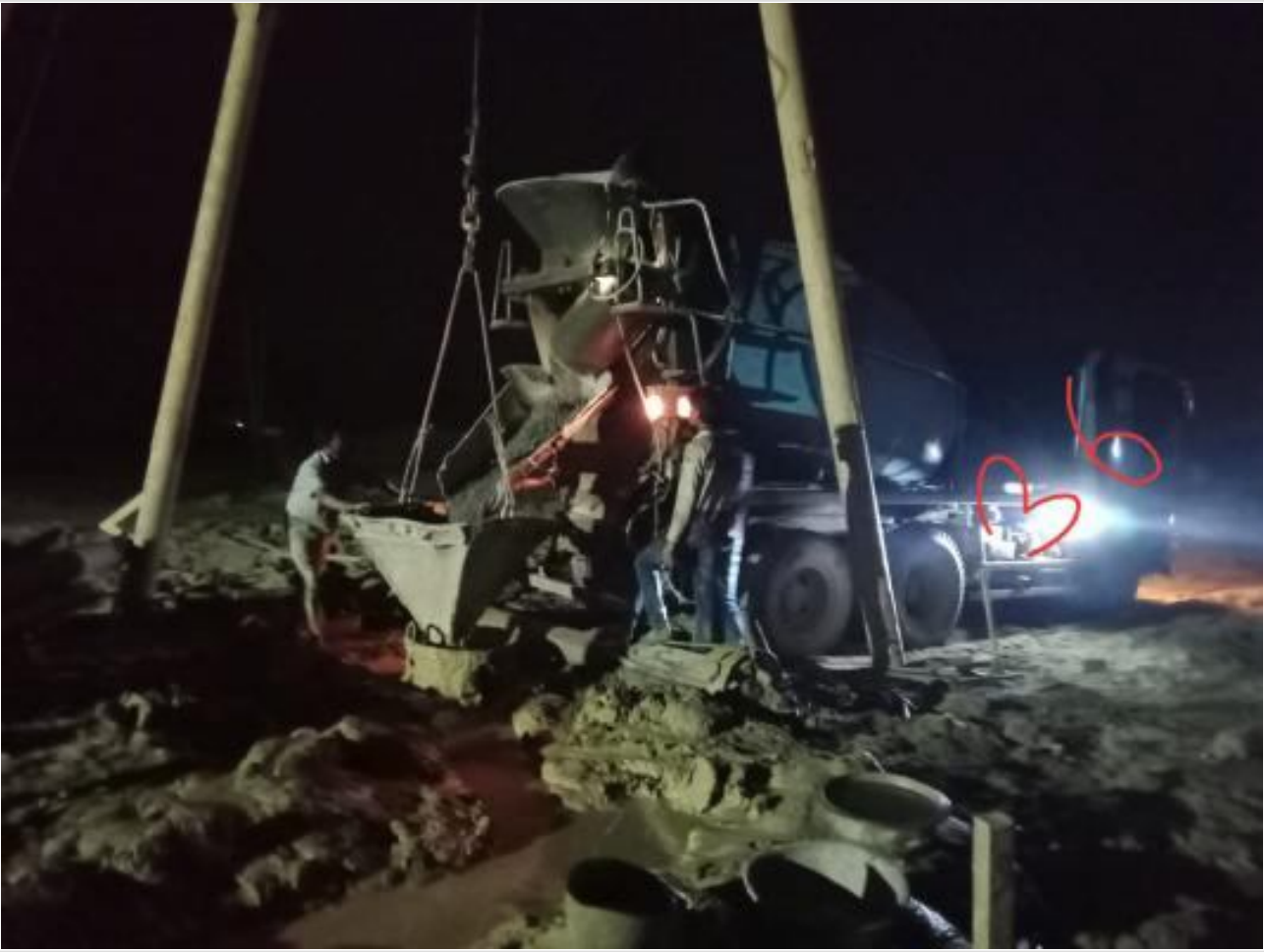
Ready mix concreting of pile on 28-02-23
