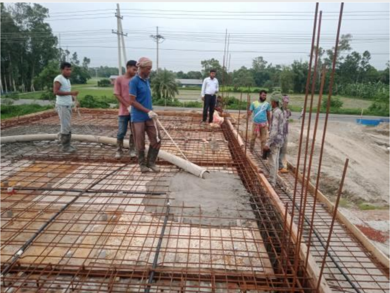
Gate House Slab casting on 11-07-23
