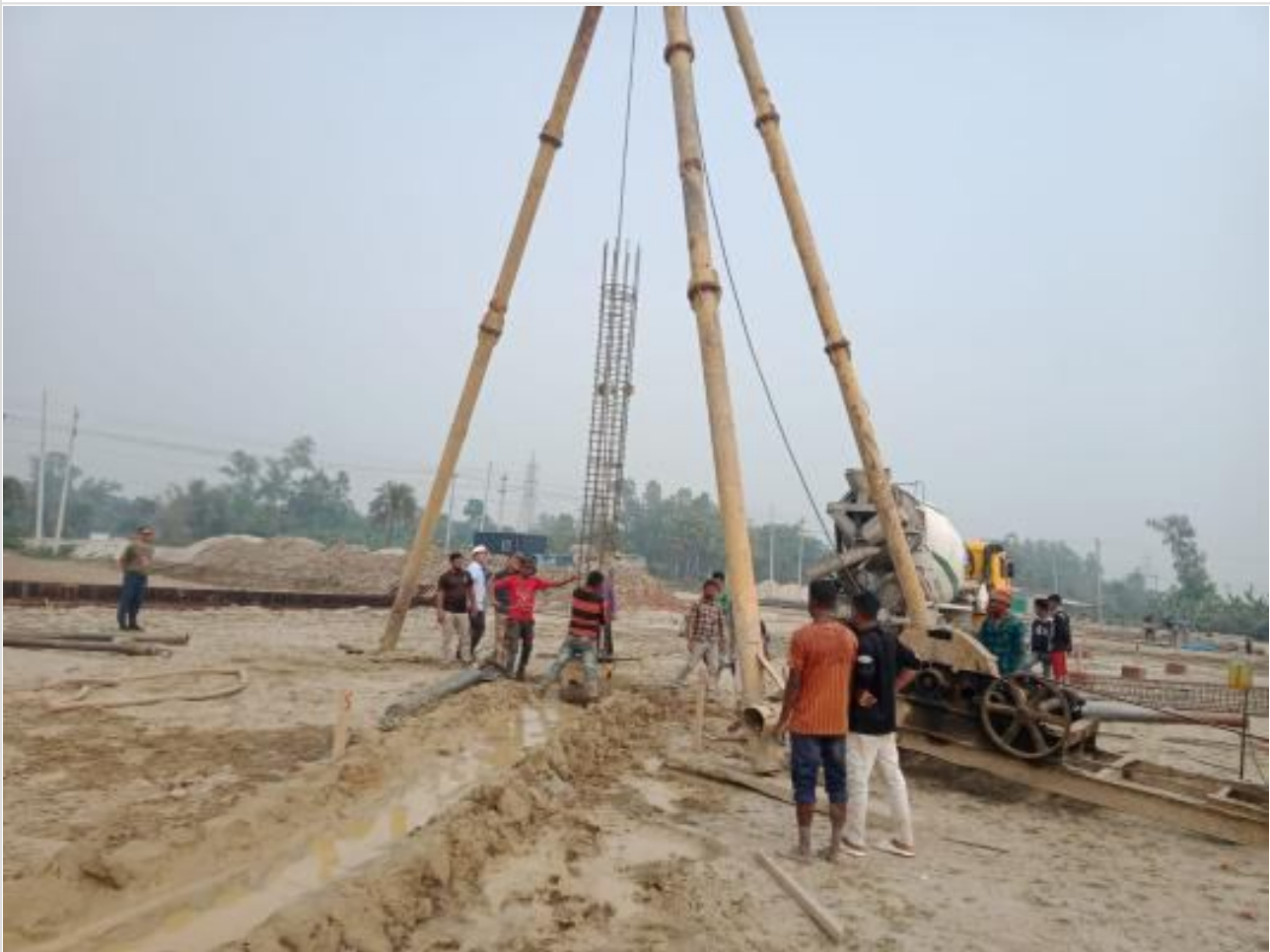
Pile Concreting on 09-02-23
