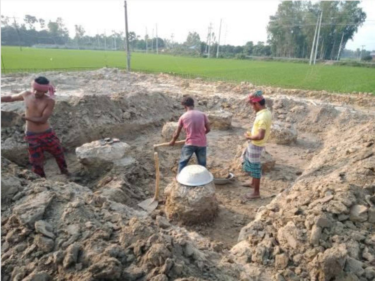
Pile head breaking on 24-03-23
