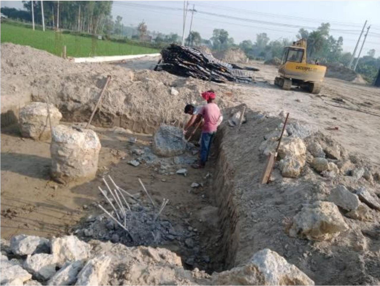
Pile head breaking on 28-03-23
