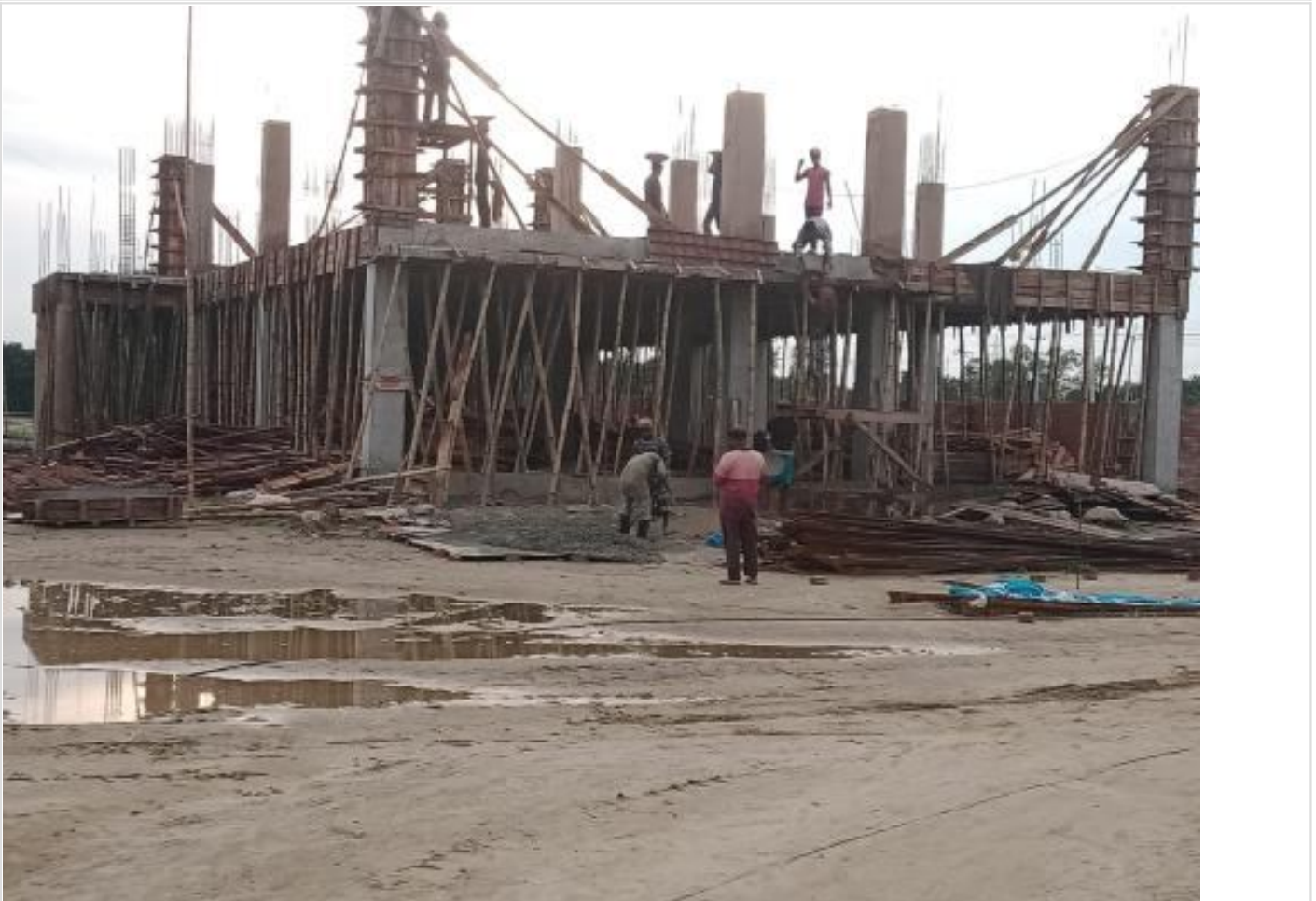
Comp. Bldg. 1st floor column work on 13-07-23
