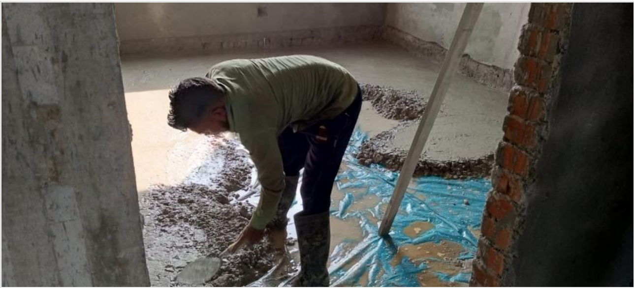
Dorm. Bldg. GF Concreting on 10-11-23
