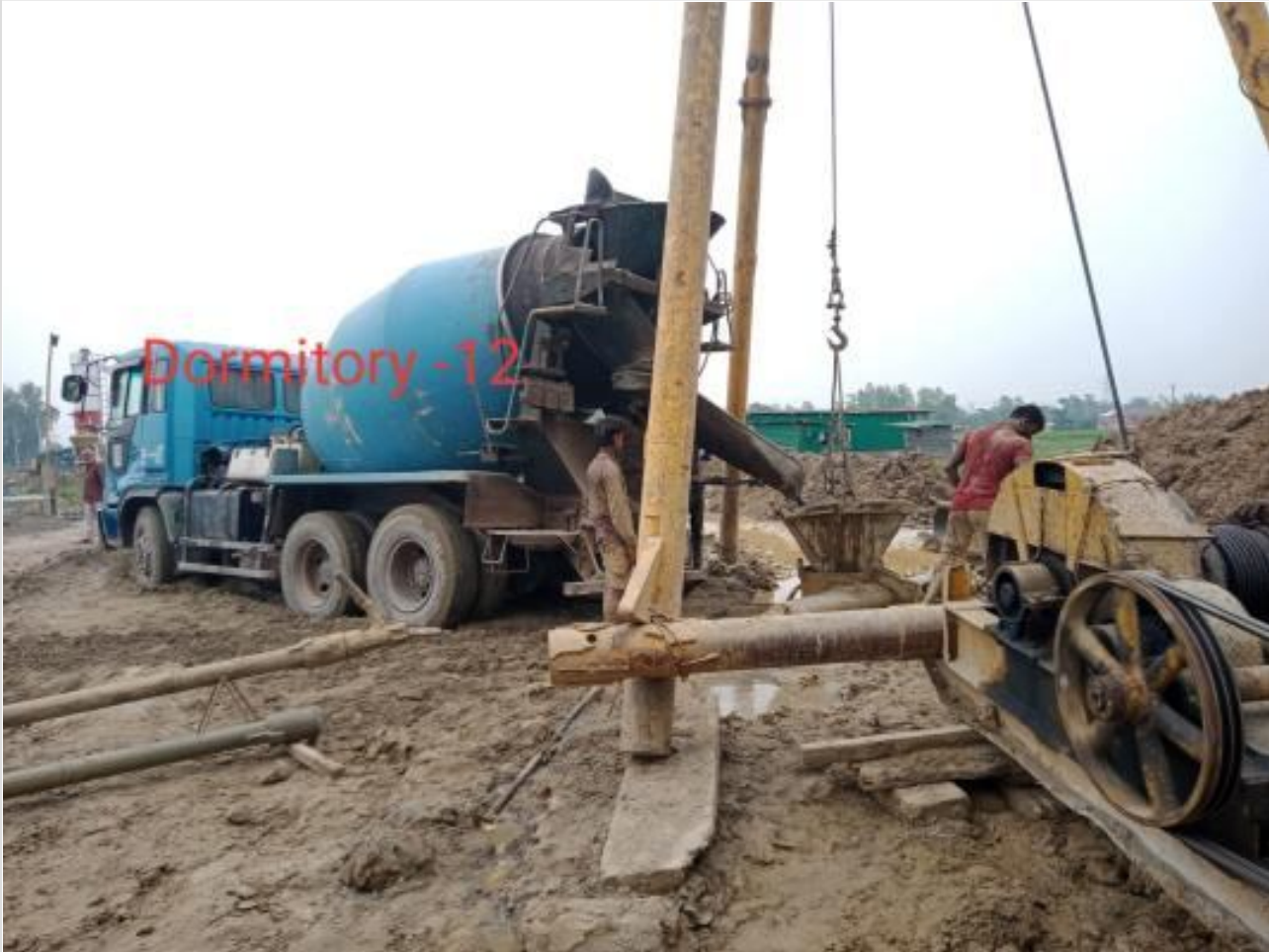
Ready mix concreting of pile on 31-03-23
