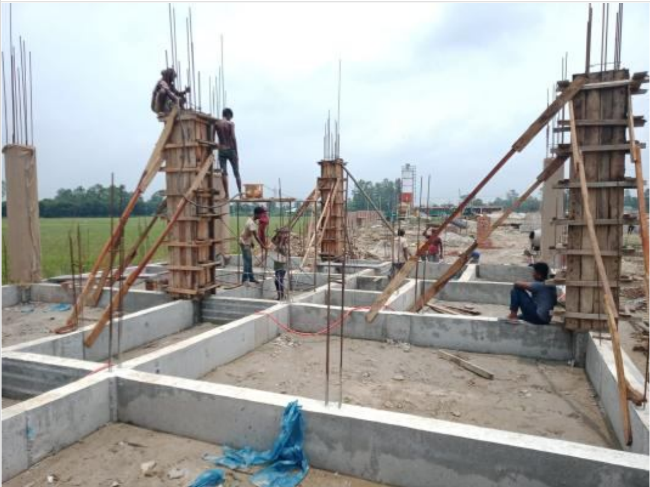
Dorm. Bldg. Column casting on 20-06-23
