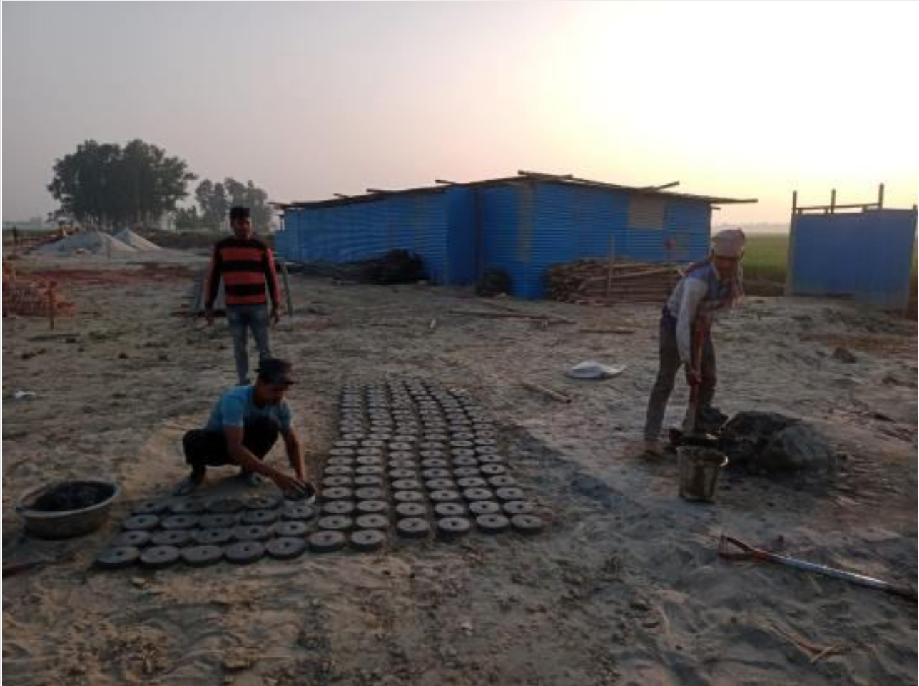
Pile re-bar spacer block making on 02-02-23
