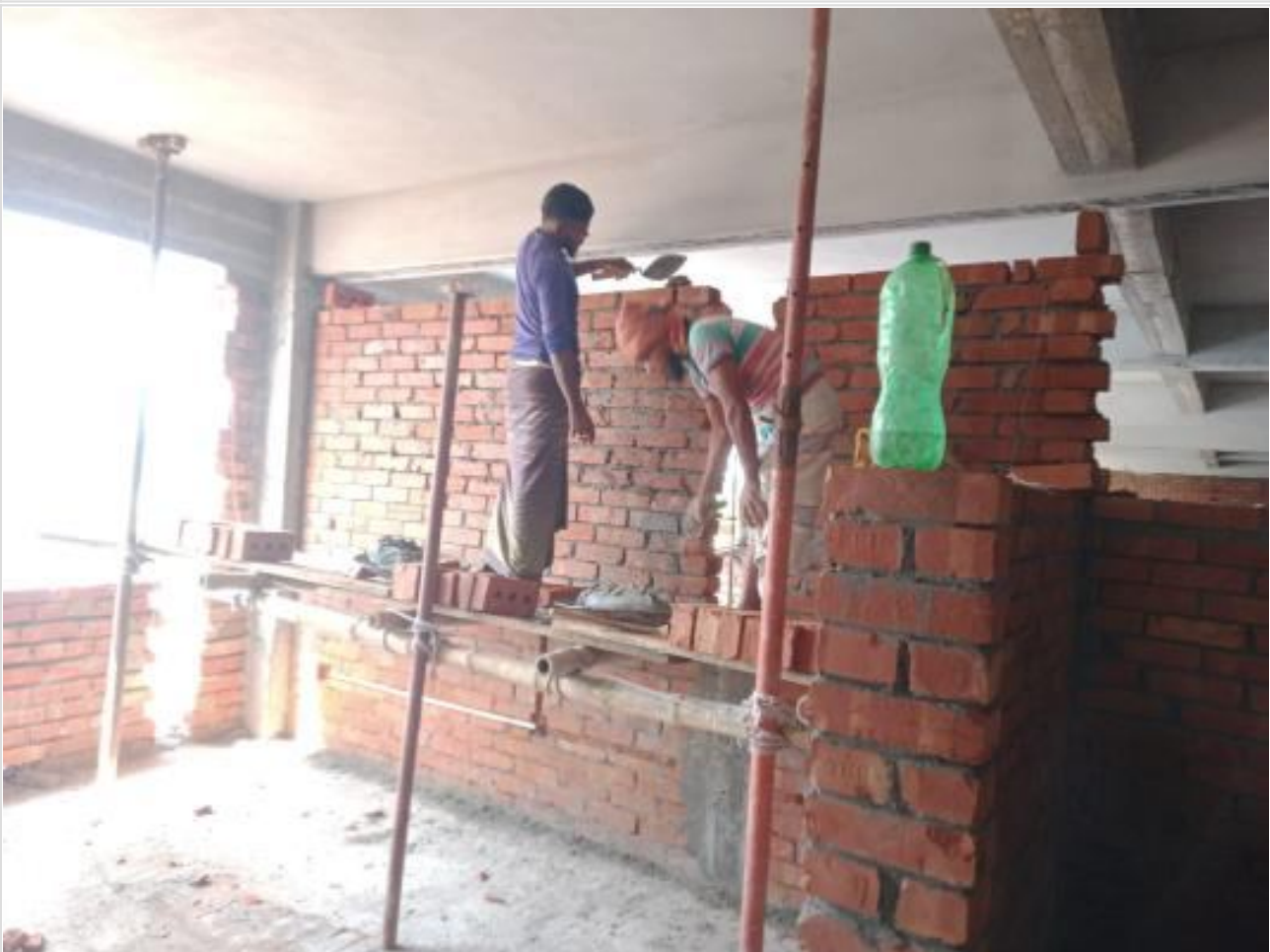
Comp. Bldg. 2nd Floor work on 10-09-23
