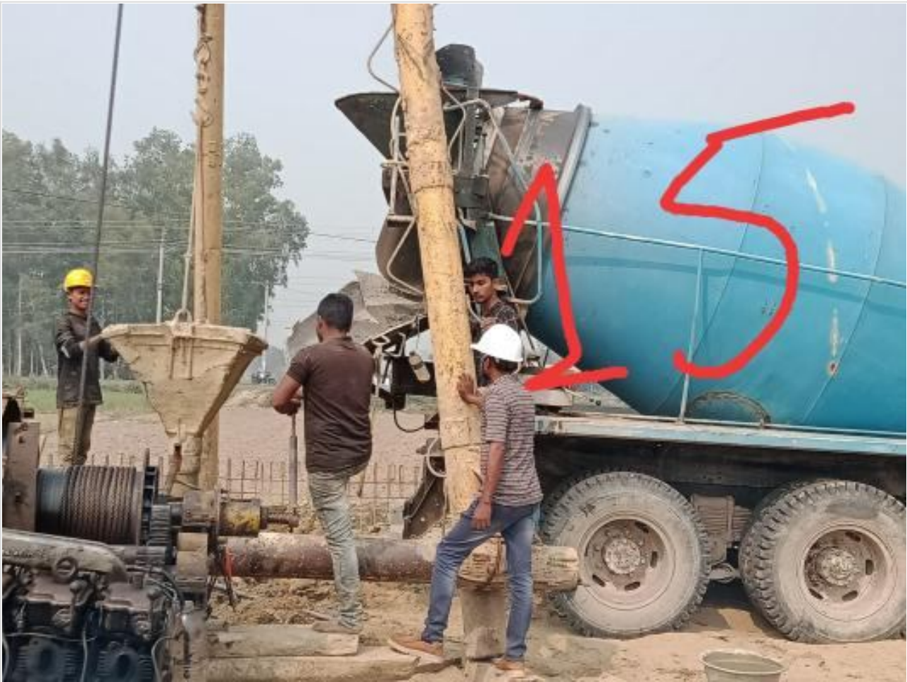
Ready mix concreting of pile on 19-02-23
