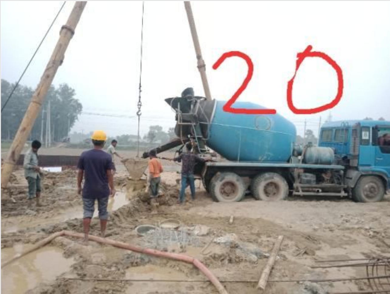
Ready mix concreting of pilewort on 22-02-23
