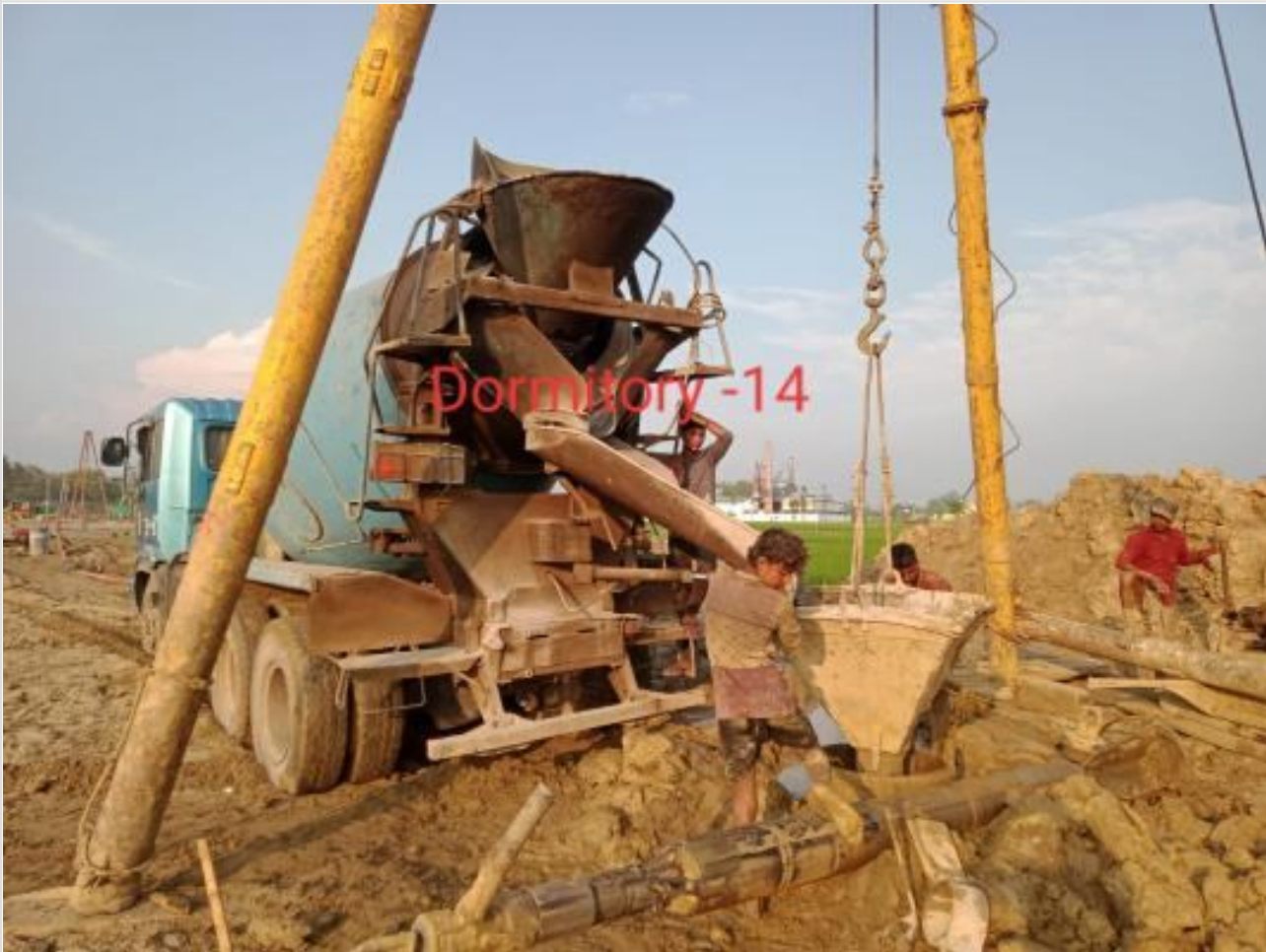
Ready mix concreting of pile on 01-04-23
