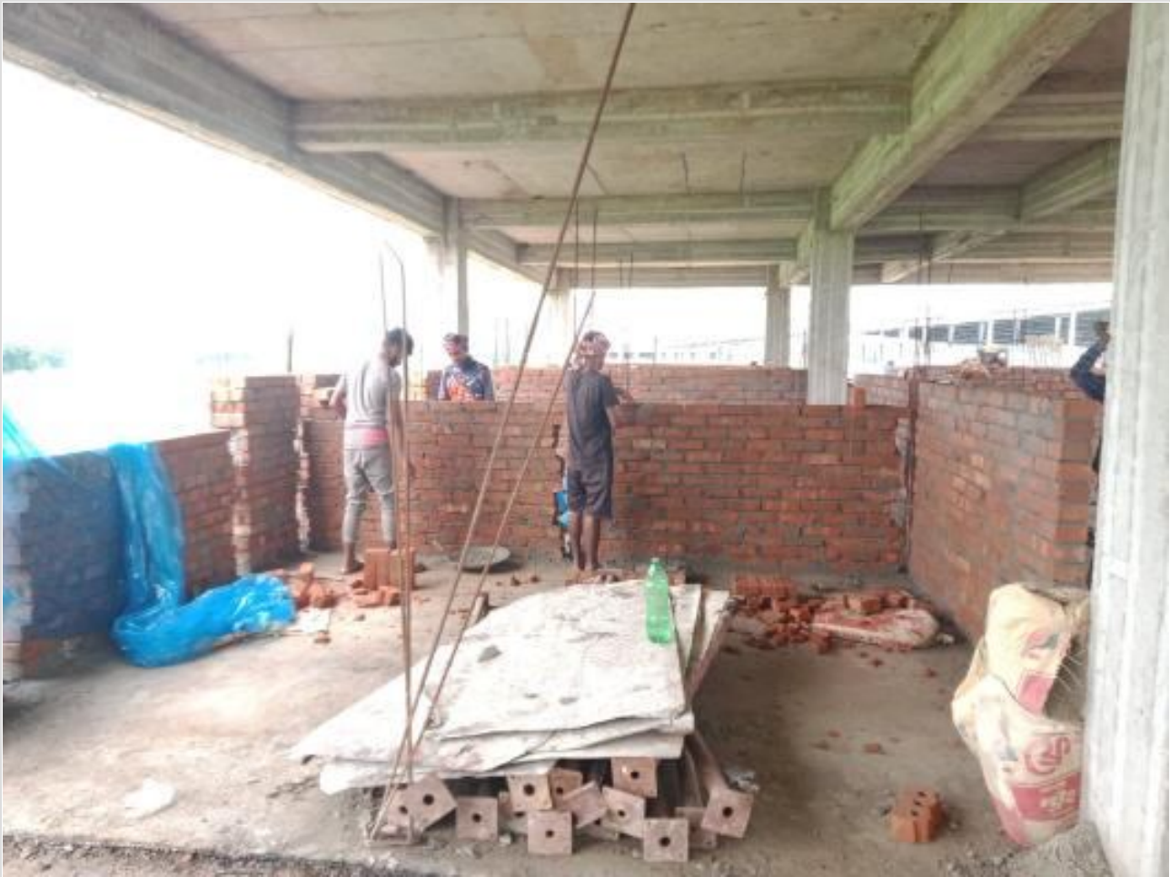
Dorm. Bldg Brick work on 07-10-23
