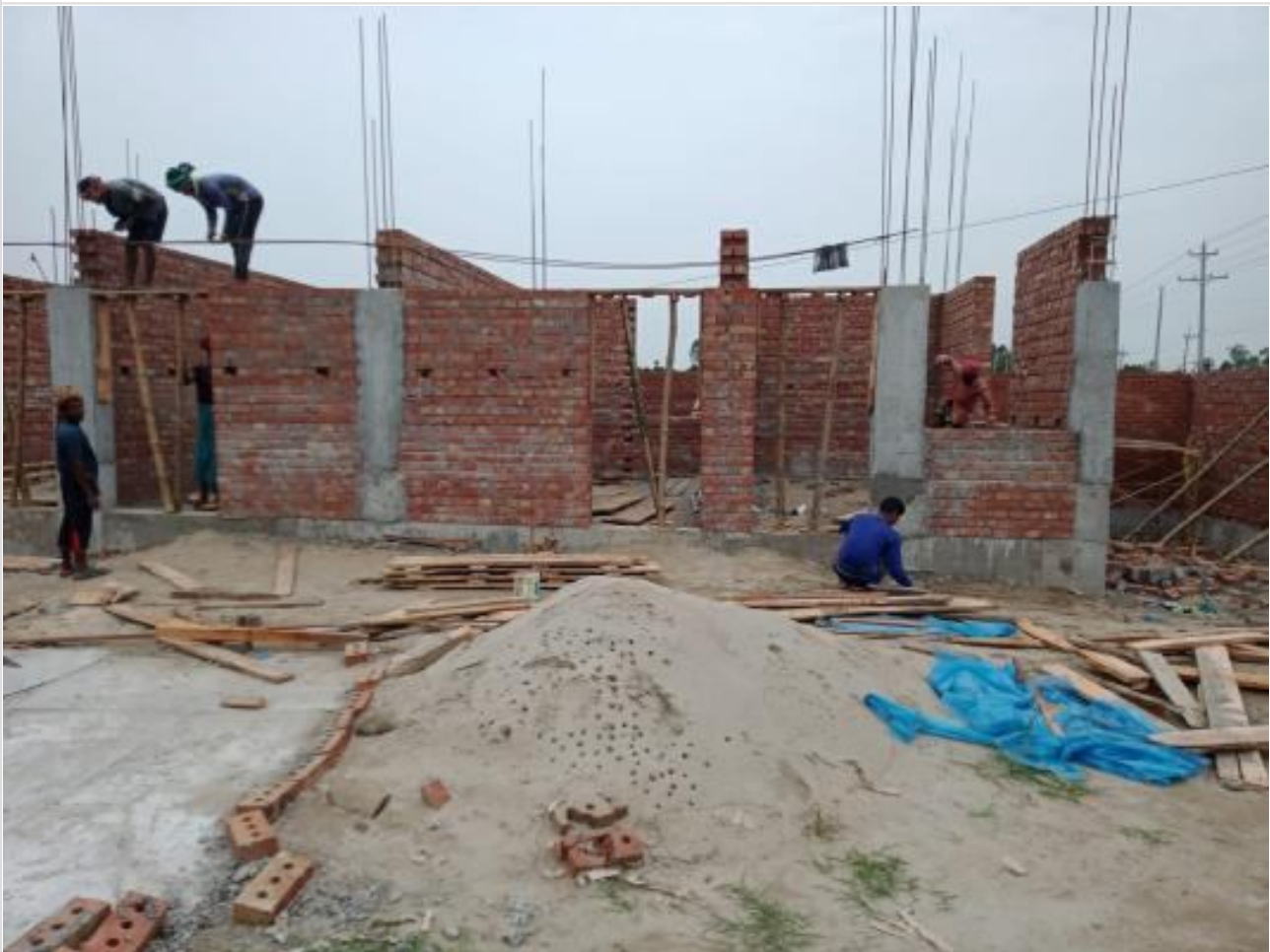
Gate house work on 19-06-23
