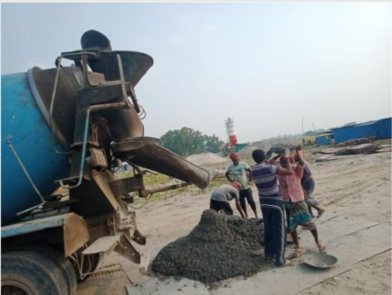
Comp. Bldg. GB casting work on 16-05-23
