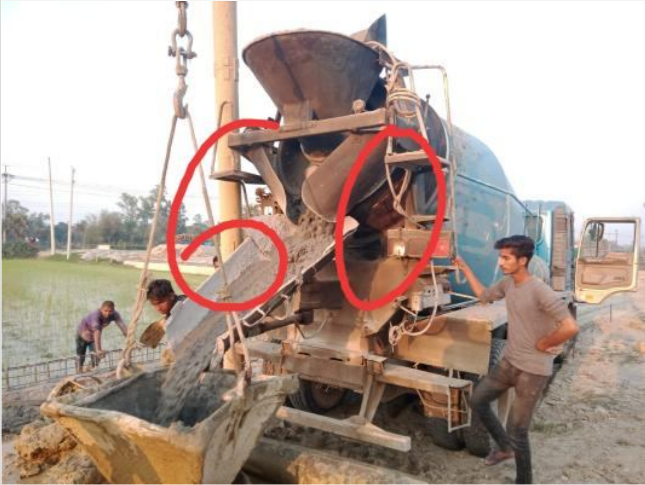
Ready mix concreting of pile on 13-03-23
