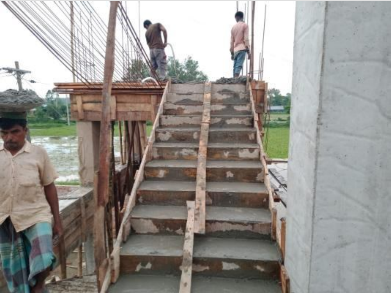
Comp. Bldg. 1st flight stair casting on 16-07-23
