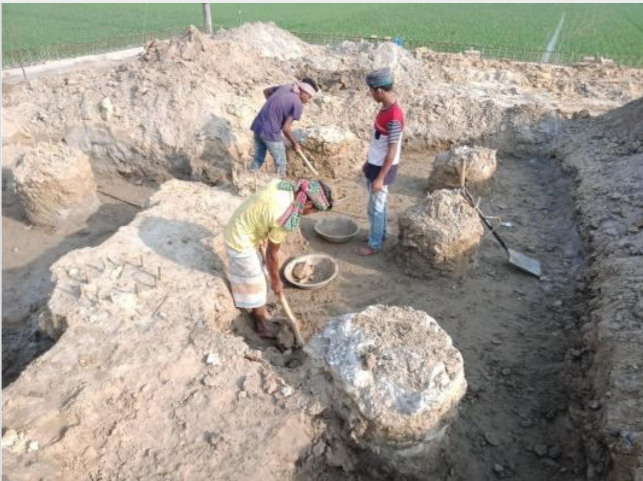
Pile cap earth cutting on 27-03-23
