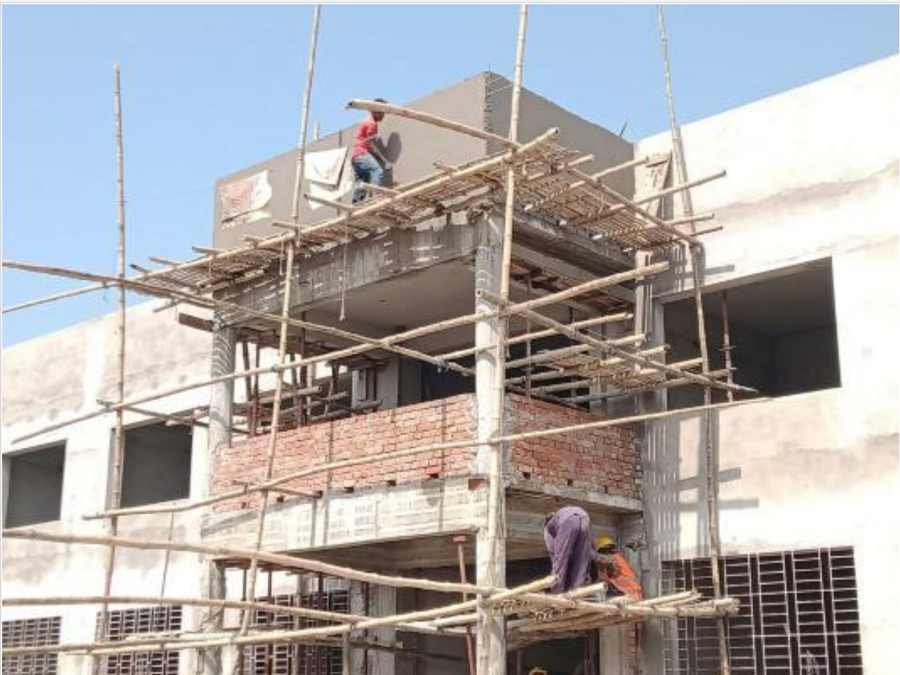
Comp. Building-Outside Plastering on 20-10-23
