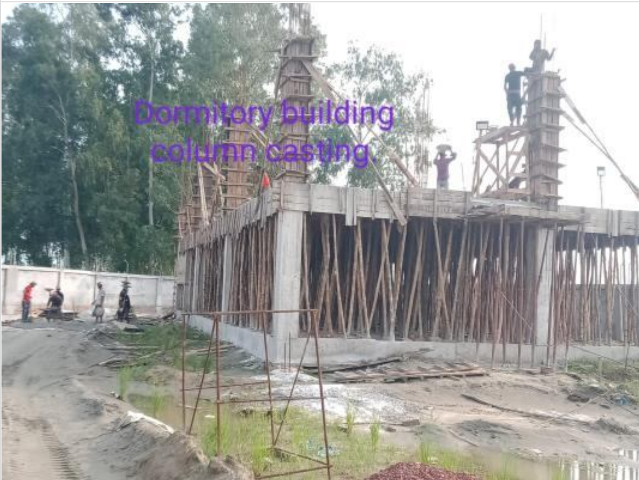
Dormitory Column Concreting on 23-08-23
