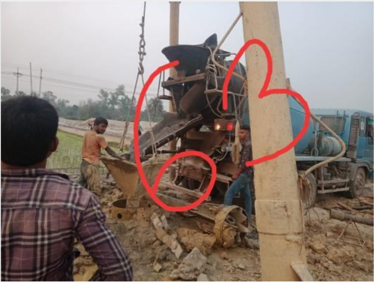
Ready mix concreting of pile on 14-03-23
