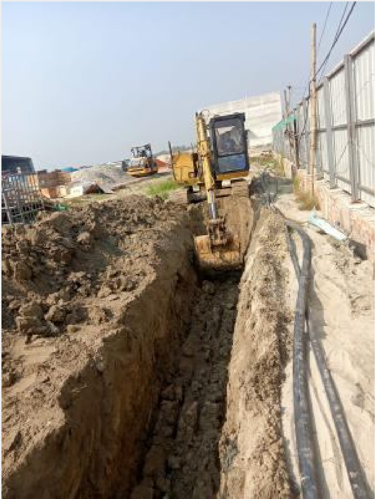
Power cable laying work on 03-11-23
