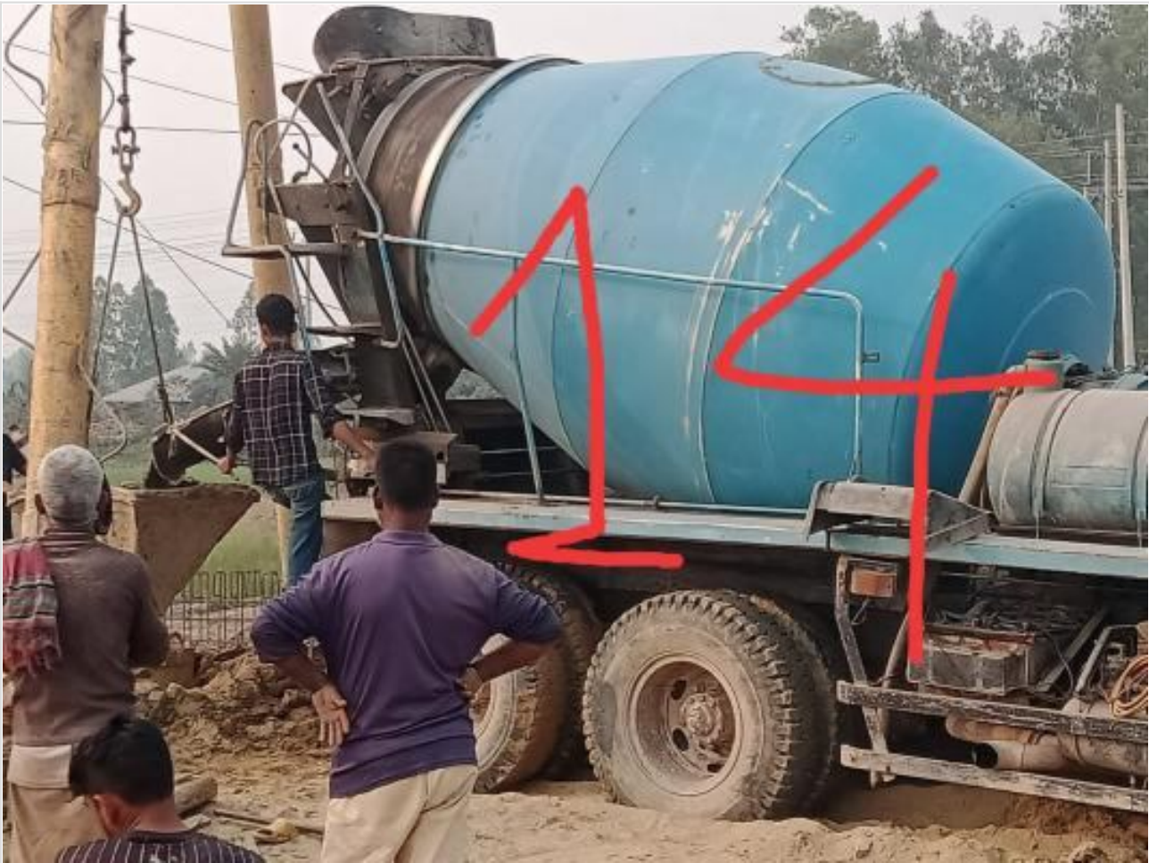
Ready mix concreting of pile on 18-02-23
