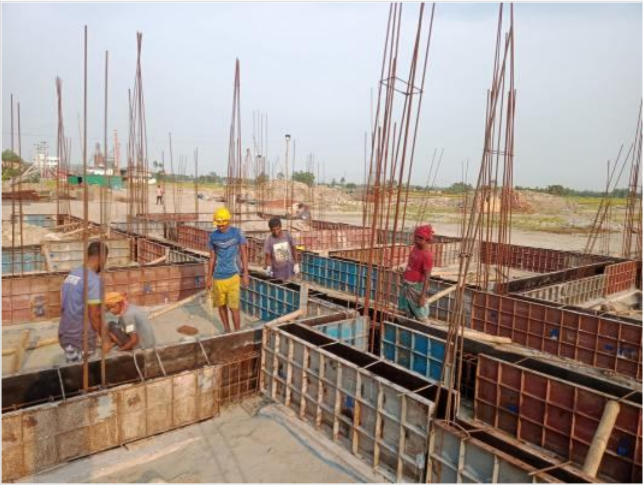
GB Shuttering work on 14-05-23
