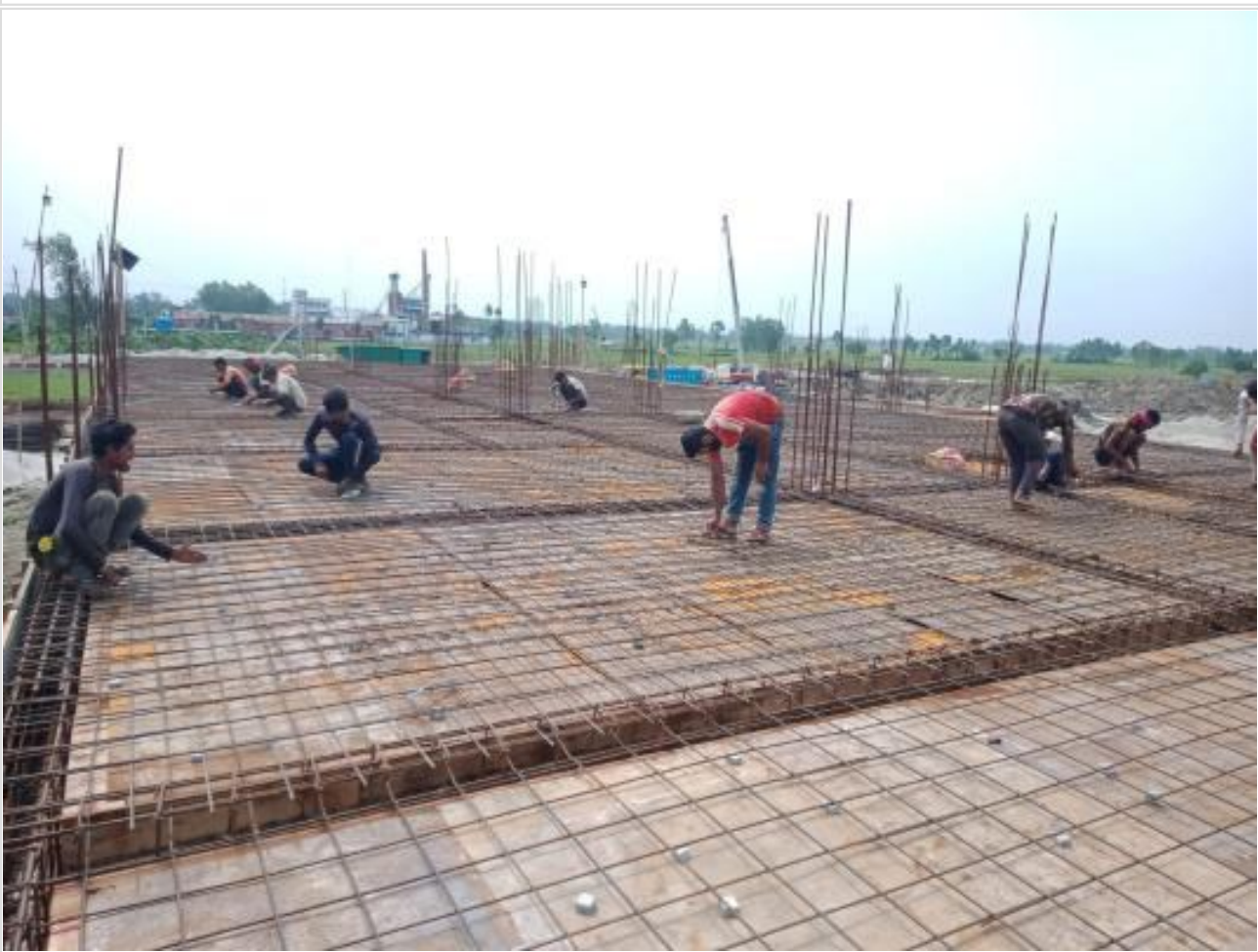
Comp. Bldg. Slab beam shuttering and rod on 19-06-23
