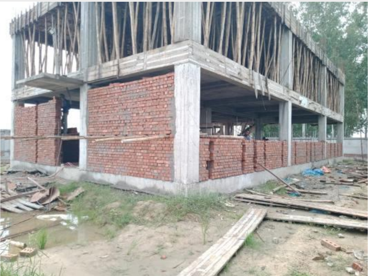
Dorm.Bldg. GF brick work on 23-09-23
