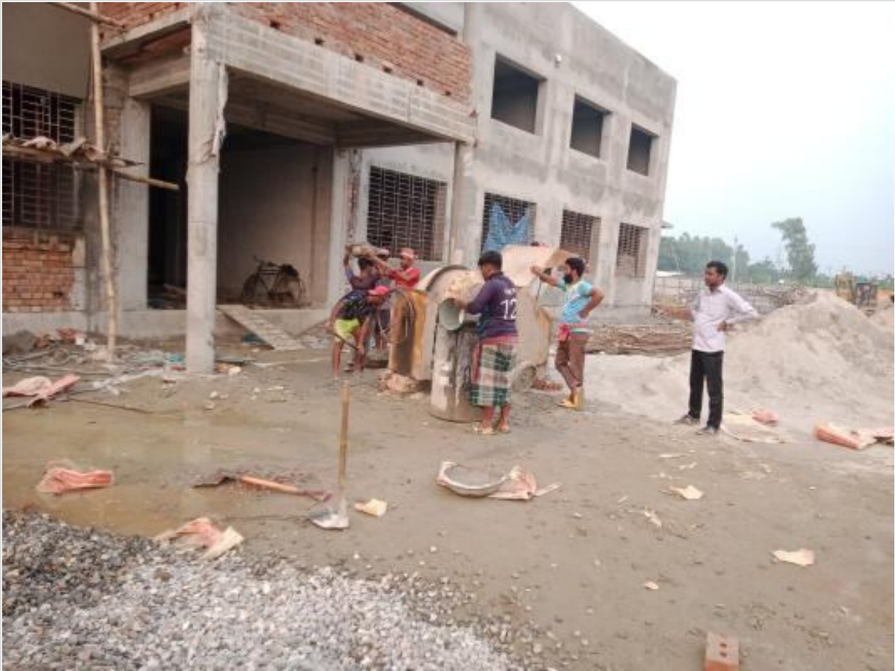
Comp. Bldg. GF casting on 16-10-23
