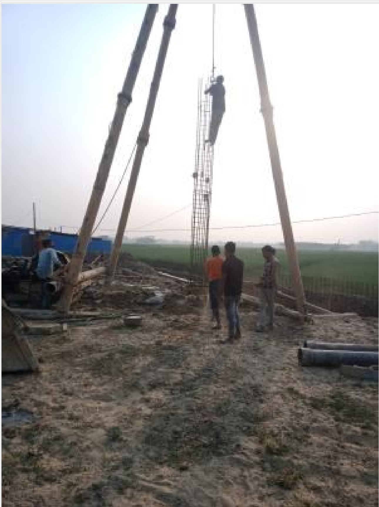
Com. Bldg. 9th pile boring on 16-02-23
