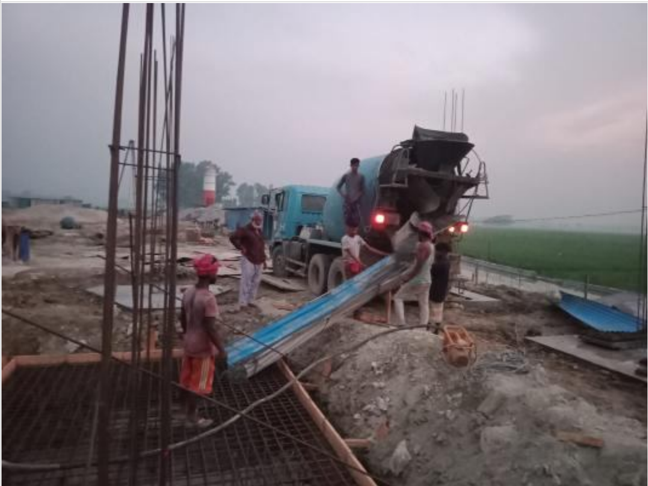
Pile Cap concreting. on 15-04-23
