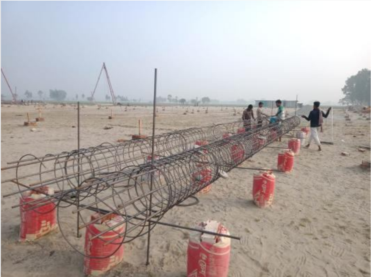
Pile Re-bar Work on 05-02-23
