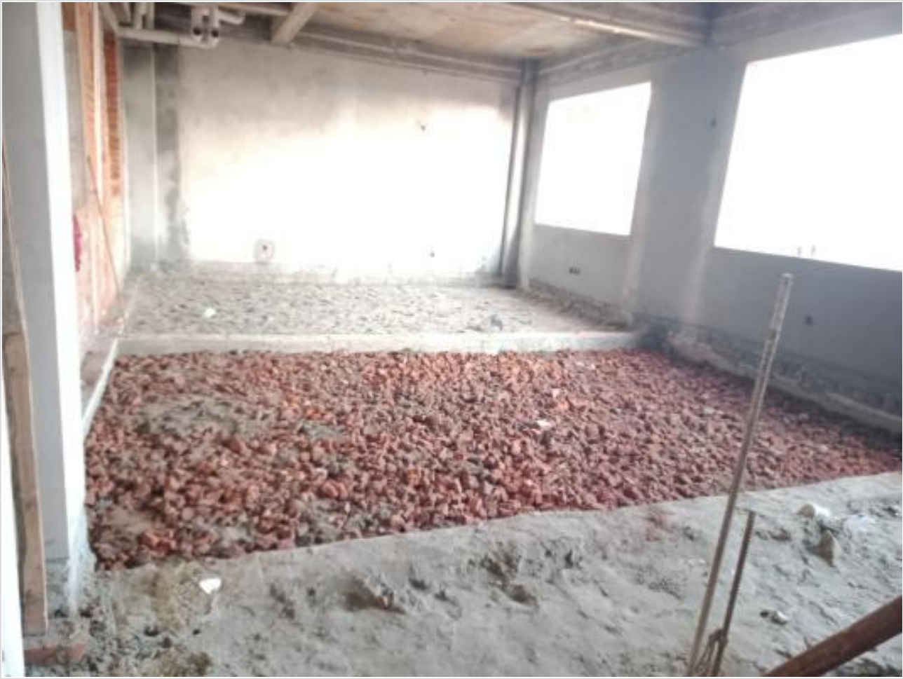
Comp. GF Cushion concreting on 15-09-23
