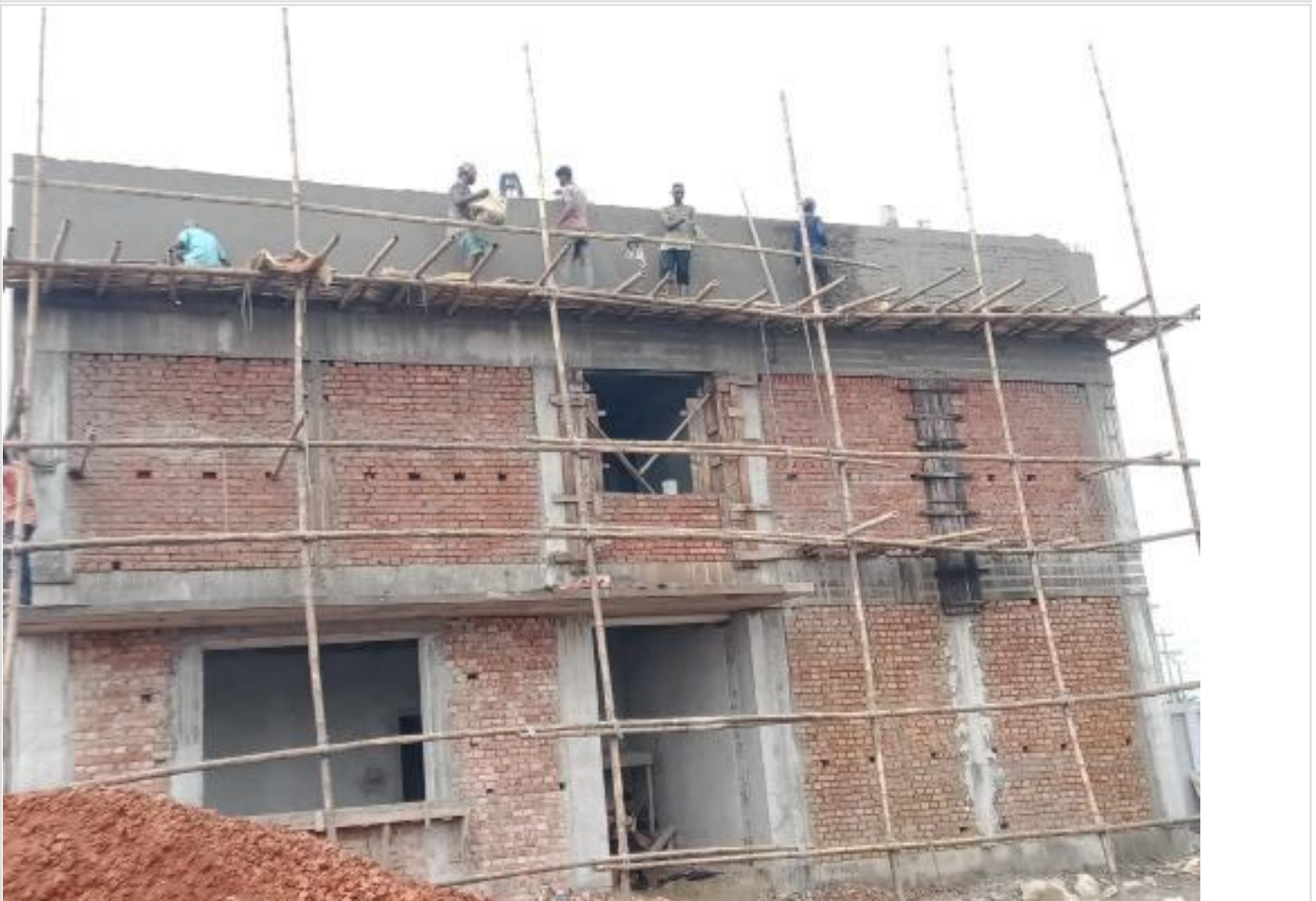
Comp. Bldg. Outside plaster work on 11-10-23
