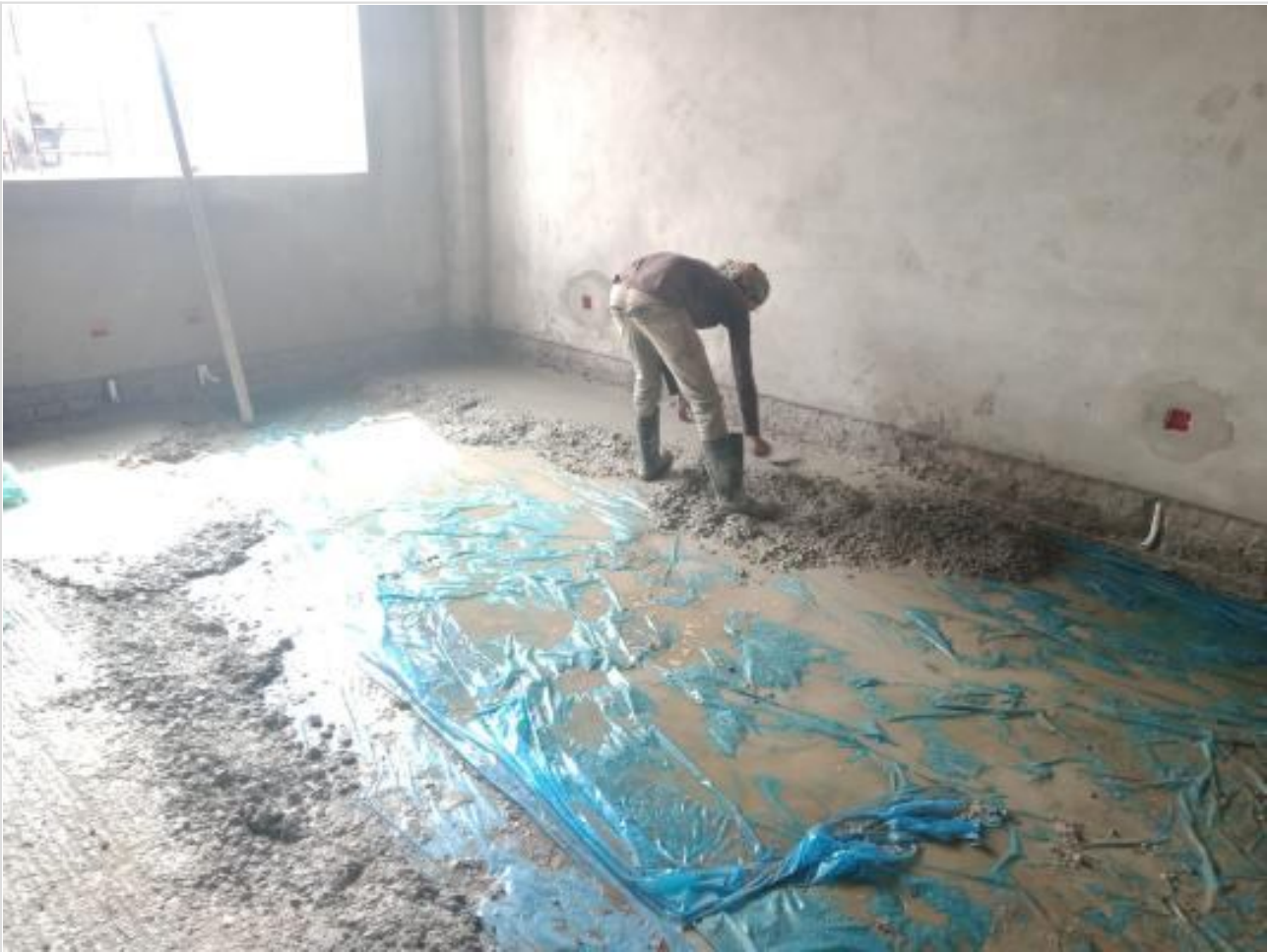
Comp. Bldg. GF casting on 09-10-23
