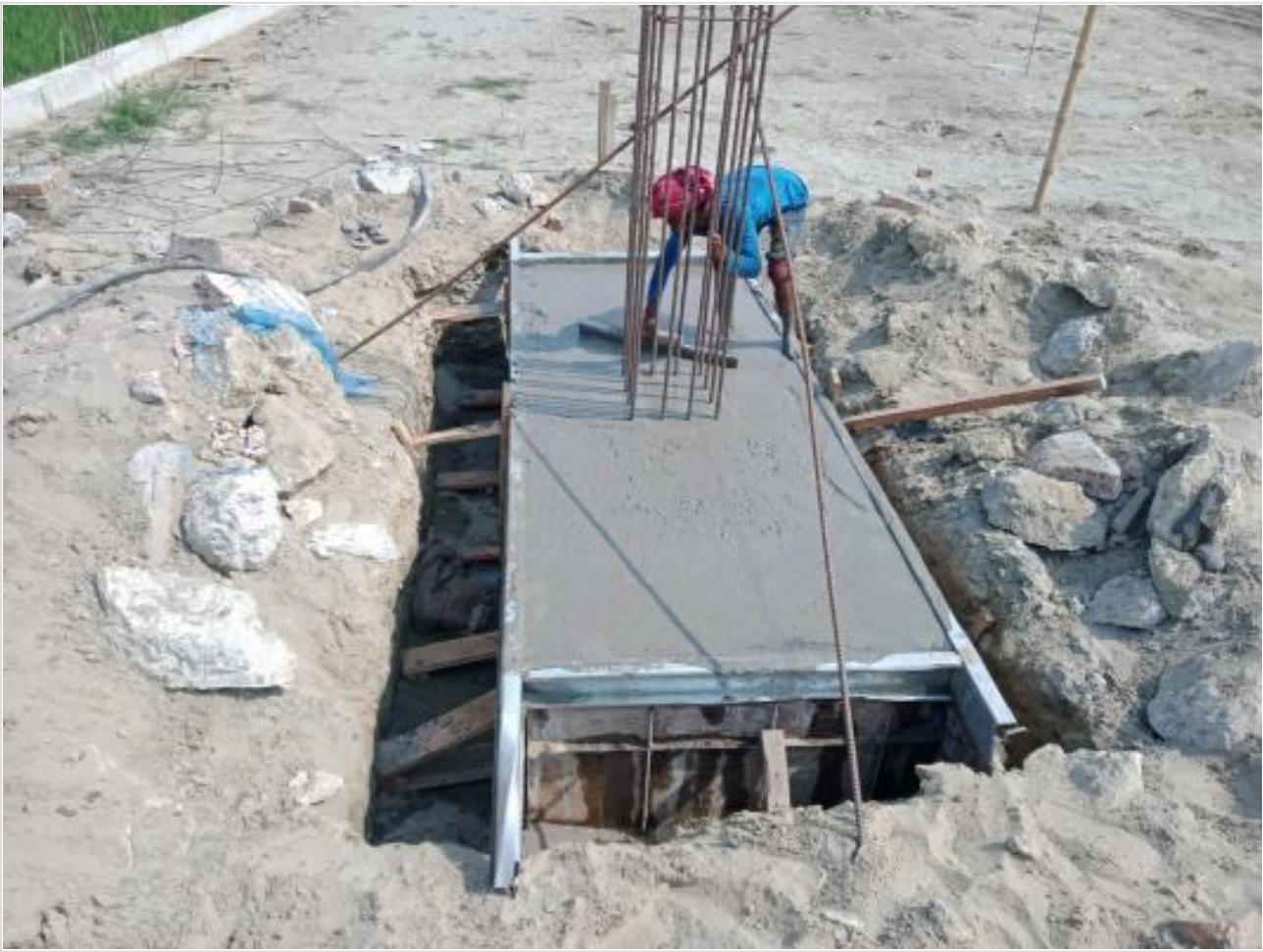
Pile cap casting on 17-04-23
