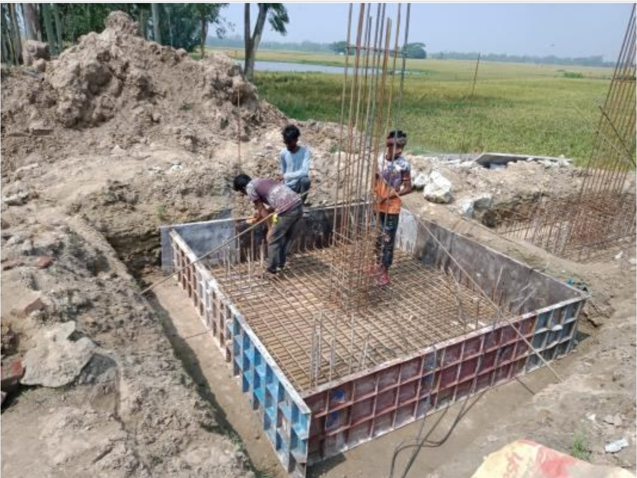
Dorm. Bldg pile cap work on 25-05-23
