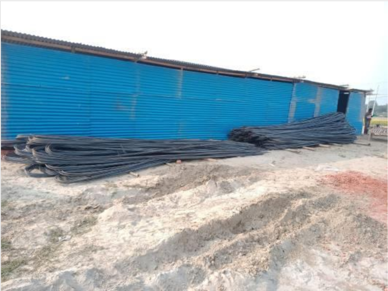
Shed completed on 22-01-23
