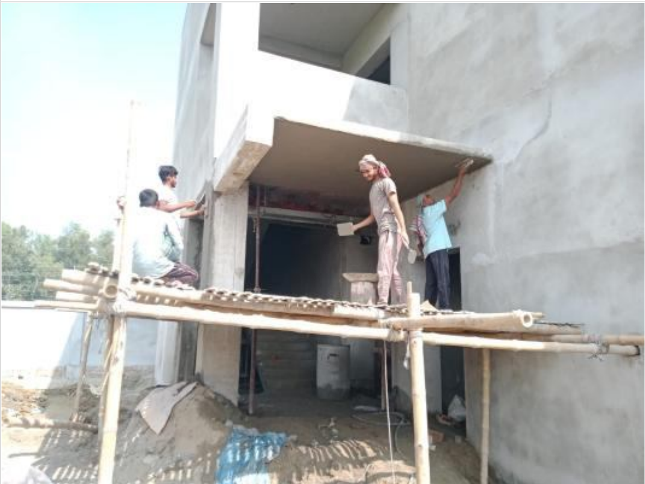
Dormitory canopy on 07-11-23
