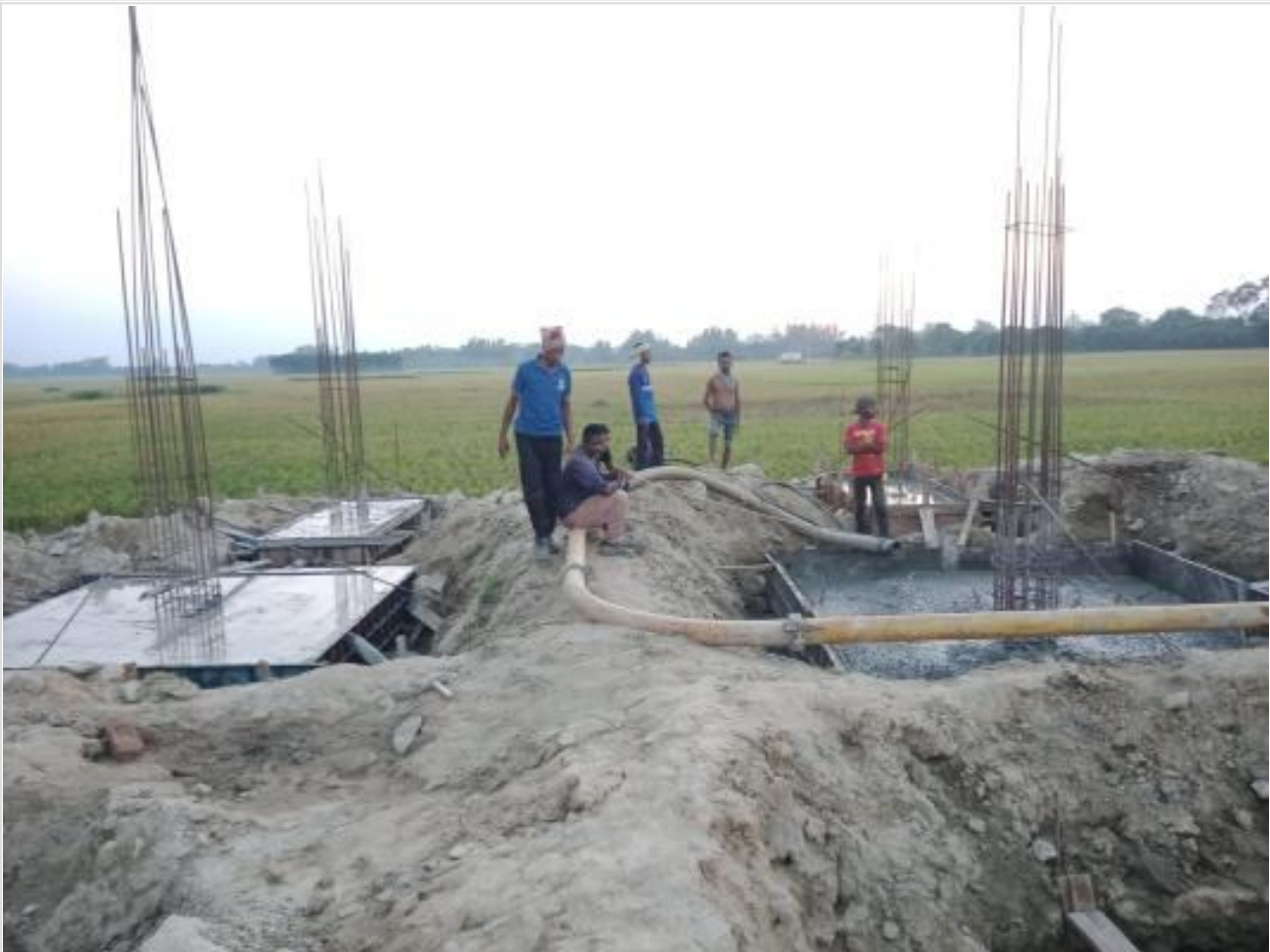
Dorm. Bldg. pile cap casting on 29-05-23
