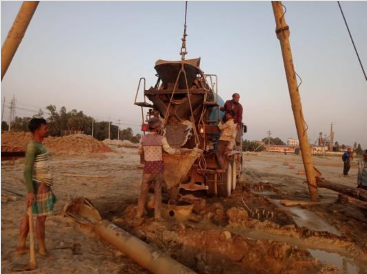
Ready mix concreting of pile on 13-02-23
