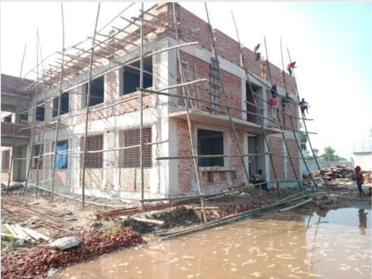
Comp. Bldg outside scaffolding on 28-09-23
