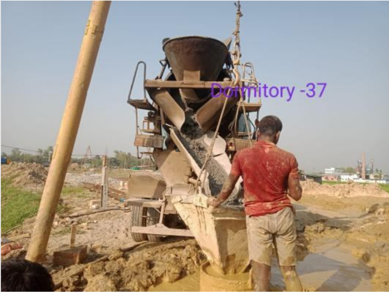
Ready mix concreting on 12-04-23
