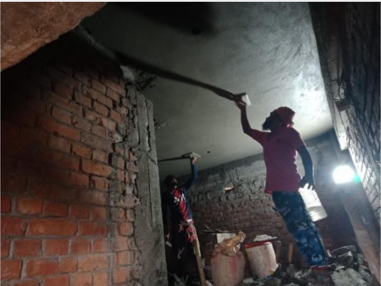
Dorm. Bldg. Ceiling Plaster on 01-11-23
