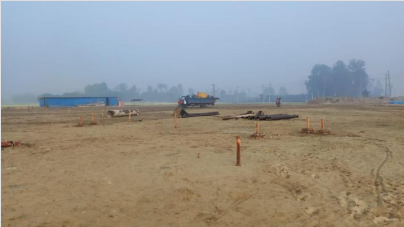
Piling Rig Mobilized on 29-01-23
