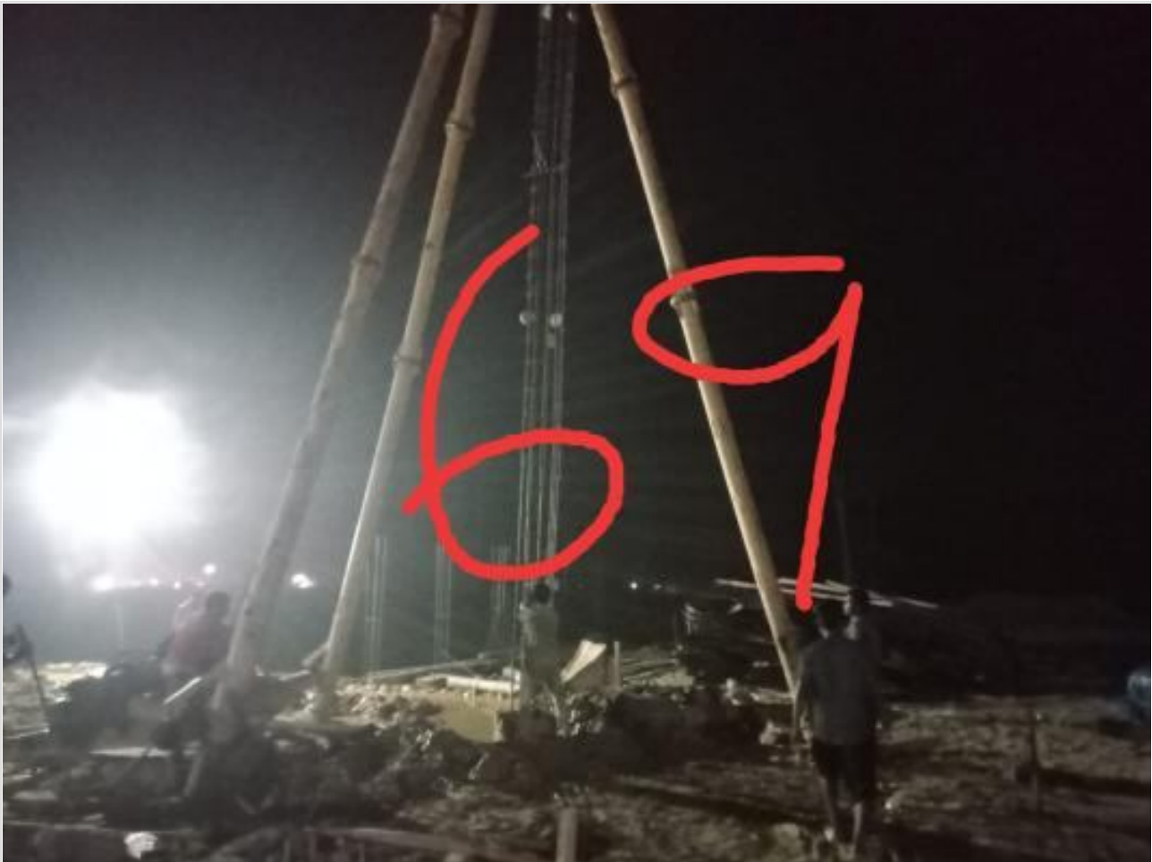
Ready mix concreting of pile on 16-03-23
