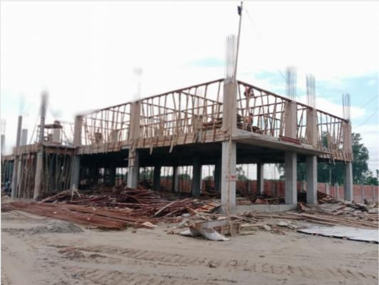
Comp. Bldg 2nd floor shuttering on 16-07-23
