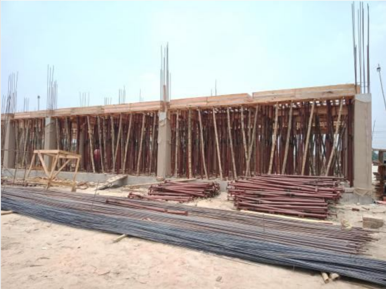
Comp. Bldg. Slab beam shuttering on 10-06-23
