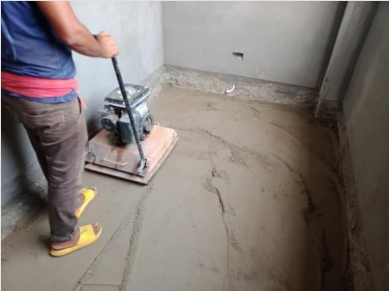
Dorm. Bldg. GF sand khoa cushion on 09-11-23
