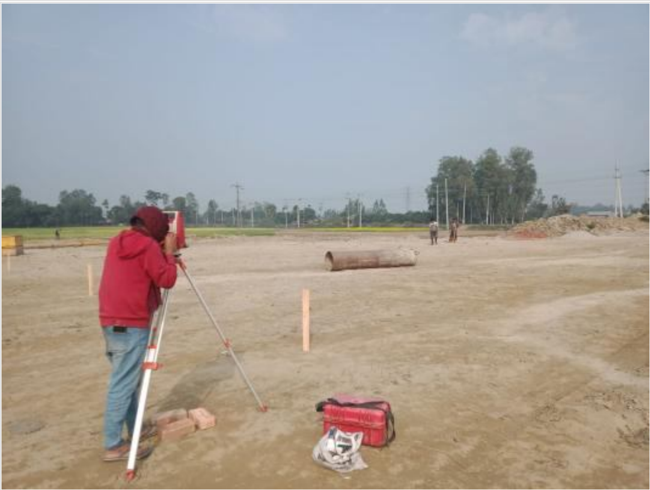
Pile Point Layout and Survey on 01-02-23
