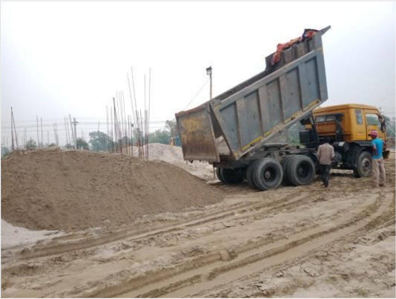
Sand filling on 21-05-23
