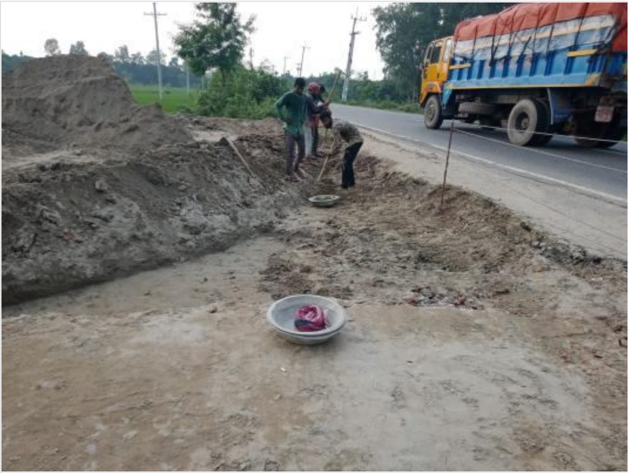
Road work on 11-10-23
