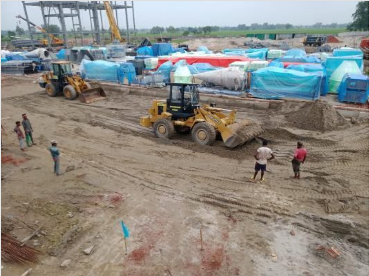
Road-Box cutting on 22-08-23
