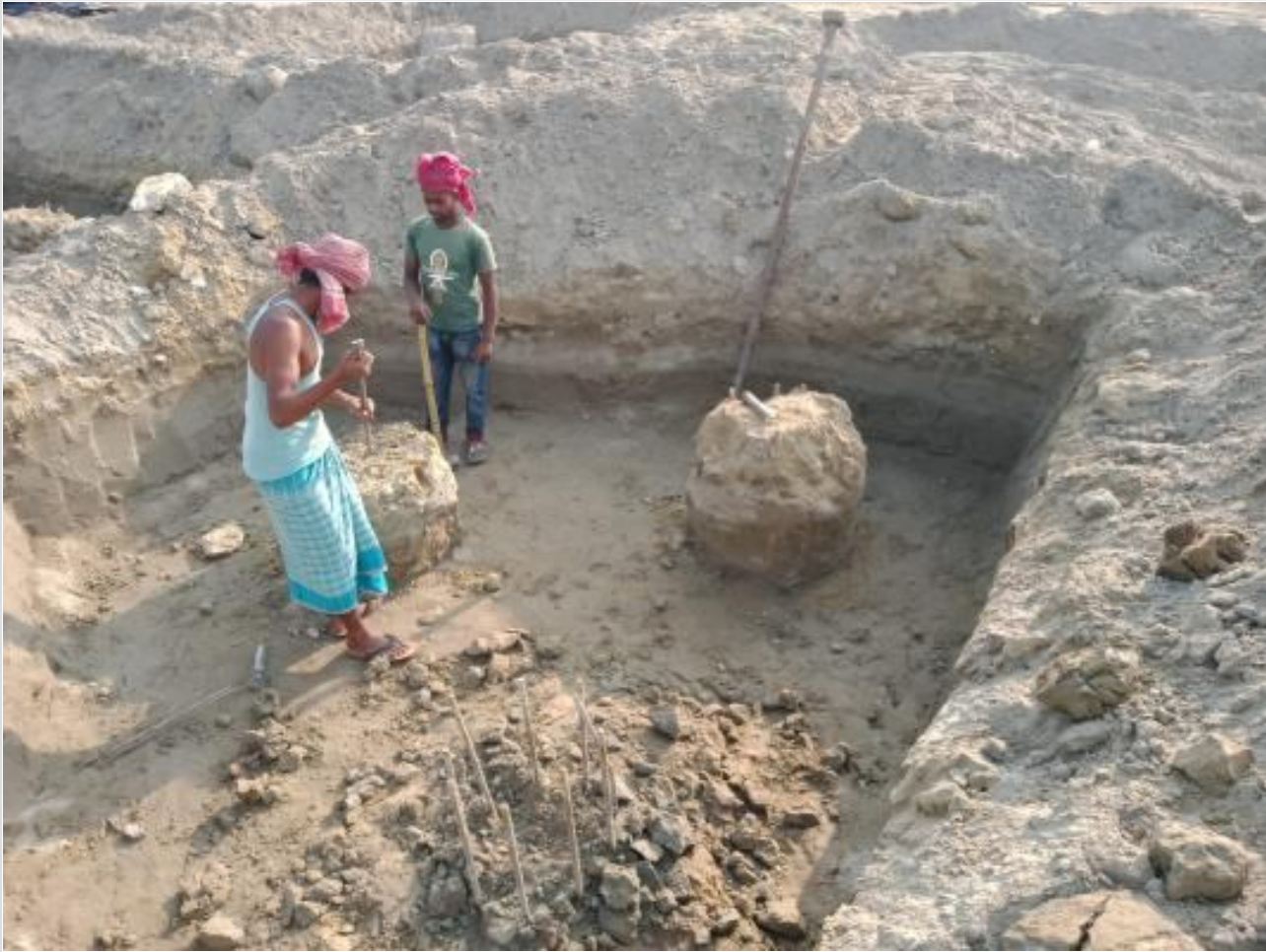
Pile cap earth cutting on 27-03-23
