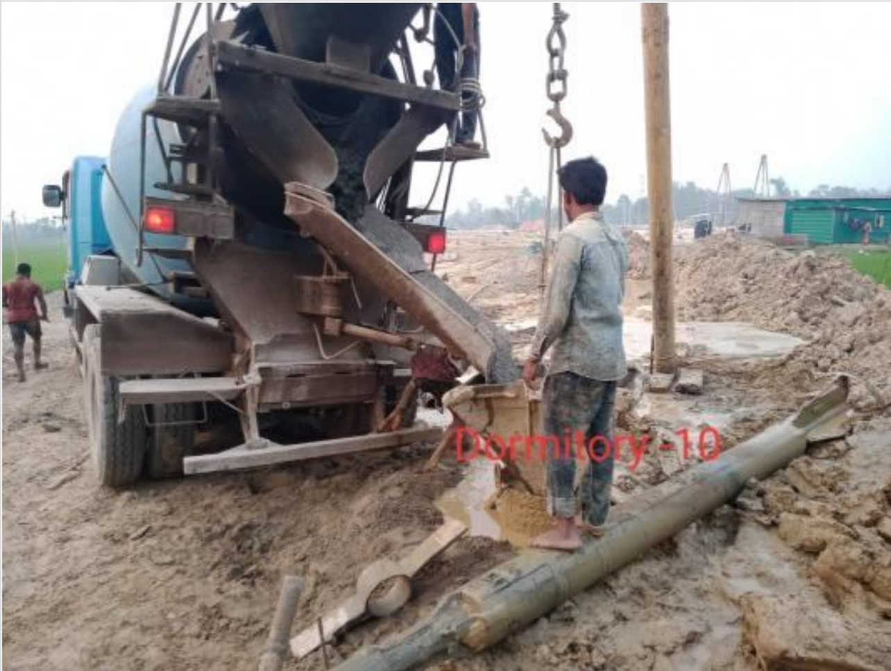
Dorm. Bldg. 10th pile concreting on 30-03-23
