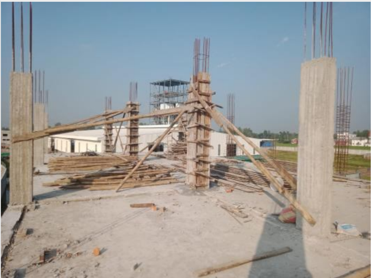
Dorm. Bldg. 2nd floor concreting work on 02-11-23
