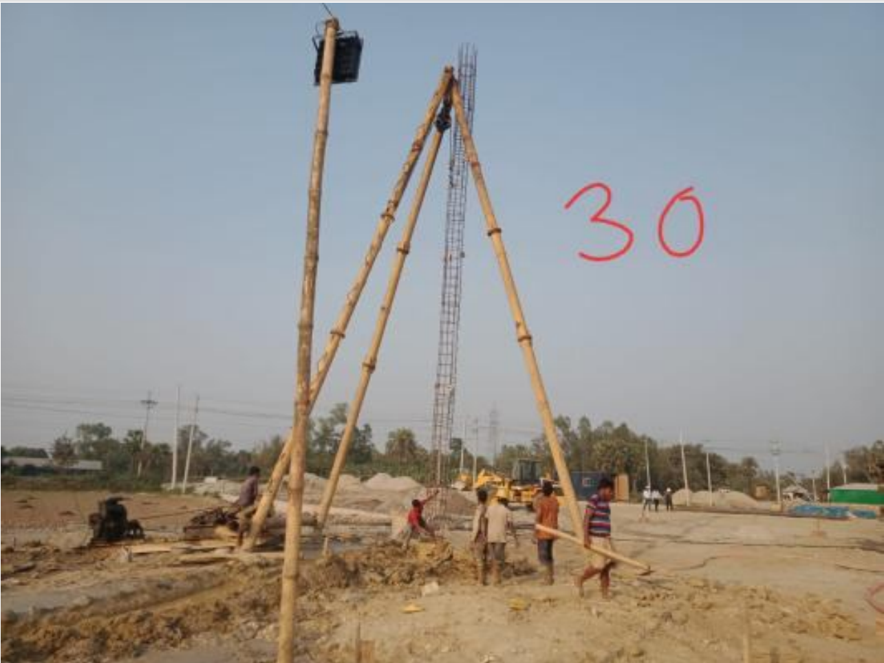
Com. Bldg. 30th pile boring on 26-02-23
