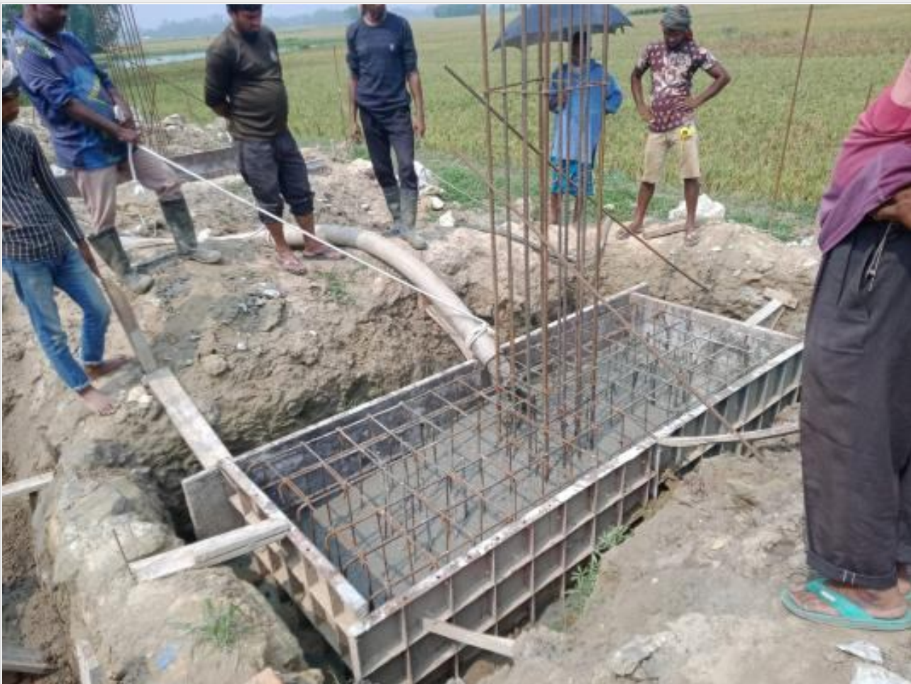
Dorm. Bldg pile cap casting on 28-05-23
