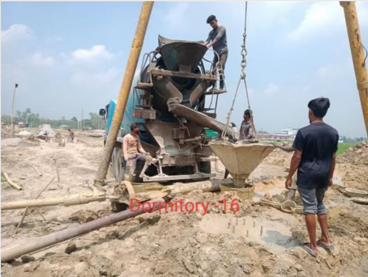
Ready mix concreting of pile on 02-04-23
