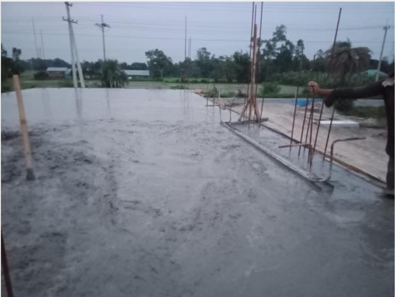
Gate House Slab Casting complete on 11-07-23
