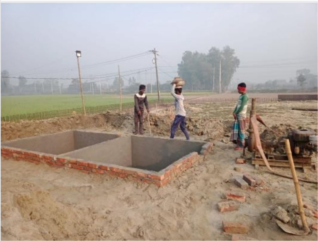
Mud Tank-1 Completed on 08-02-23
