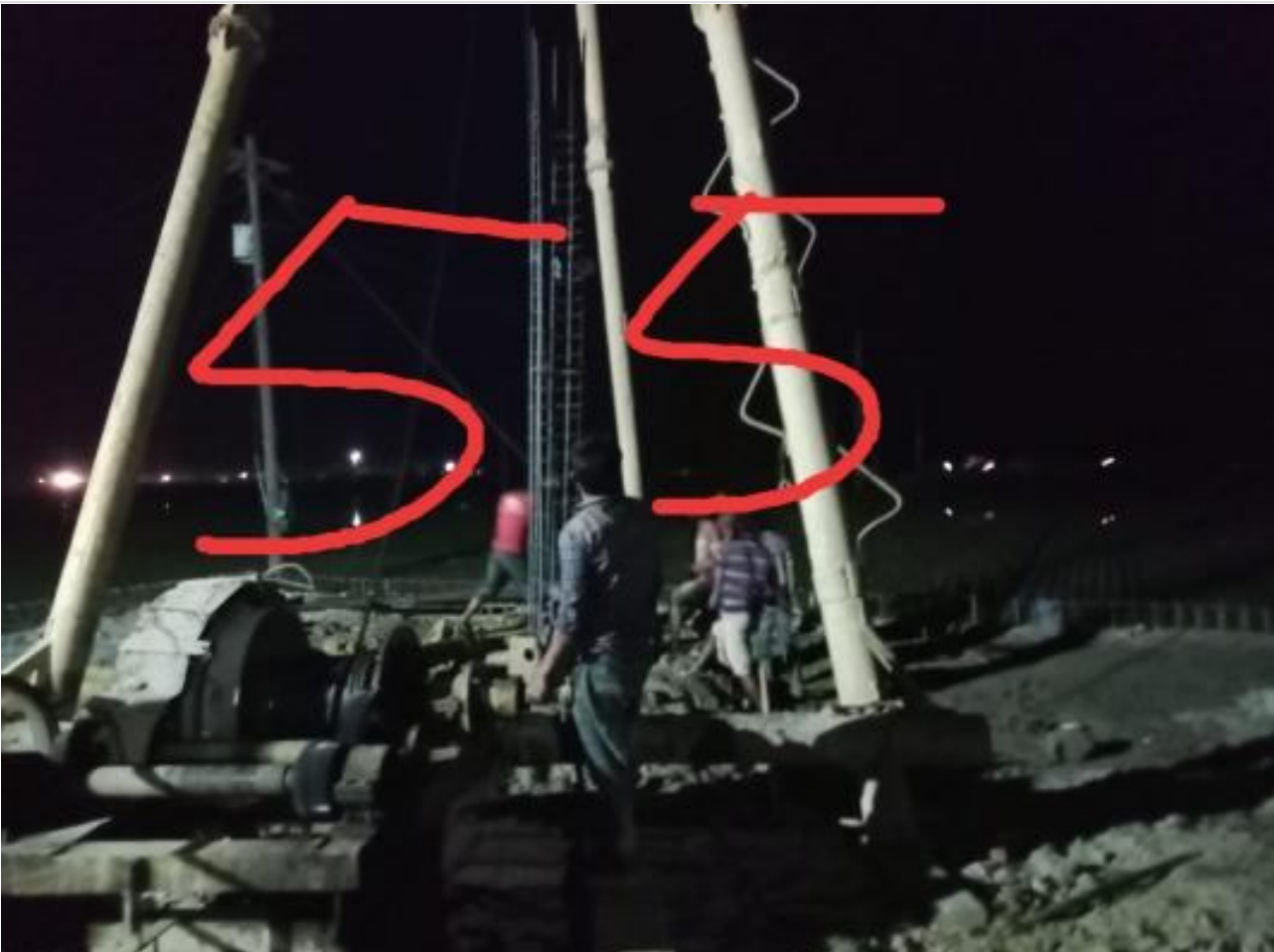
Ready mix concreting of pile on 10-03-23
