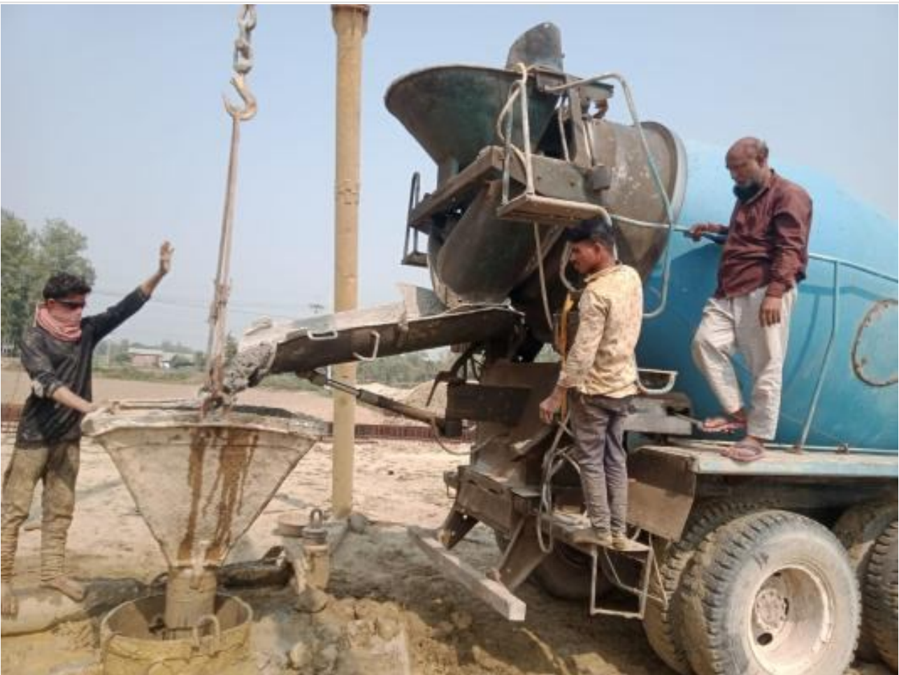
Ready mix concreting of pile on 15-02-23
