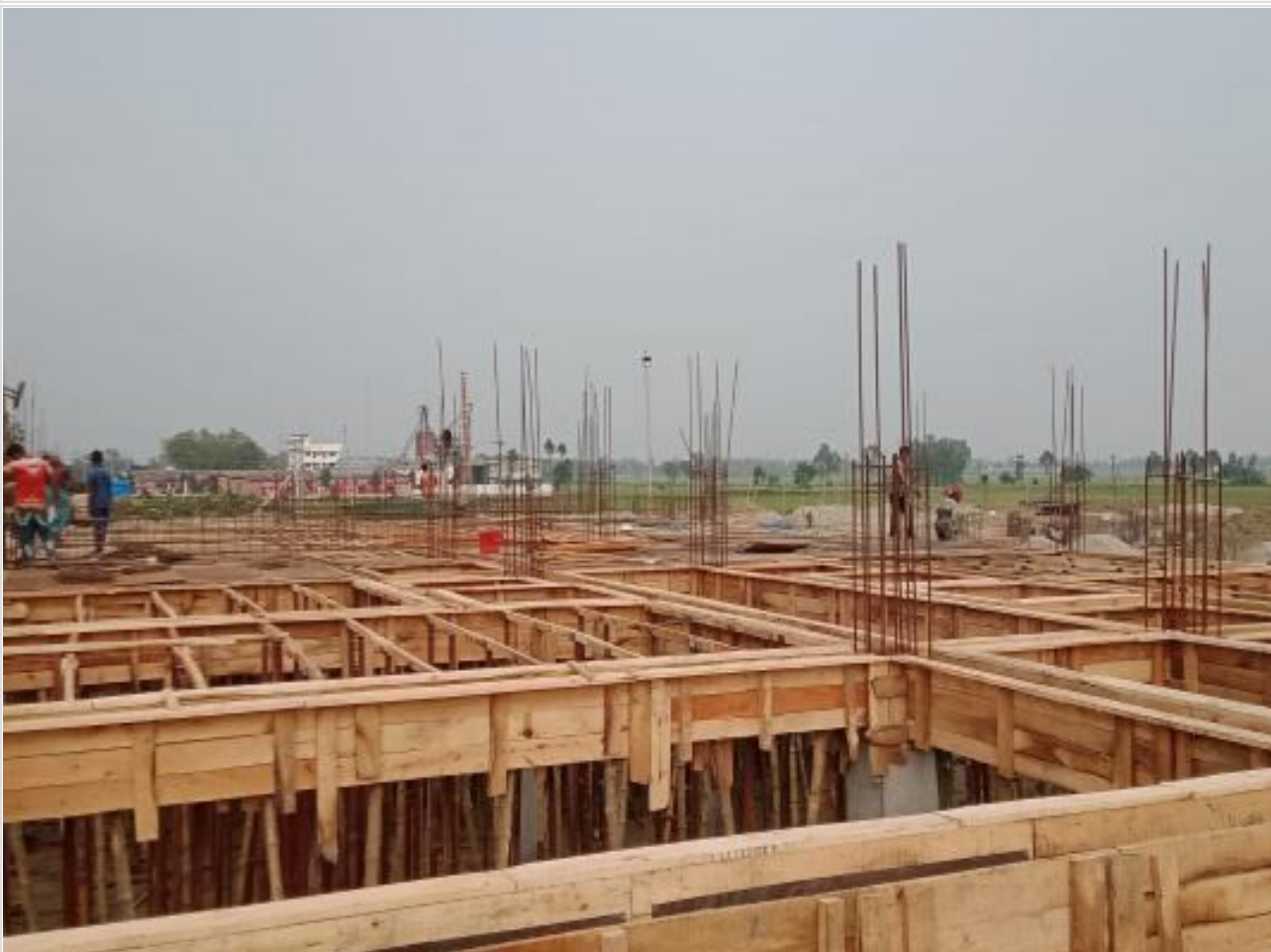
Comp. Bldg. Slab beam shuttering on 10-06-23
