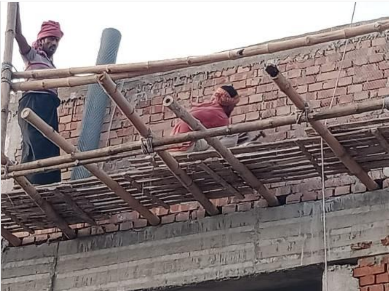
Comp. Bldg. Prepared for Out side plaste on 08-10-23
