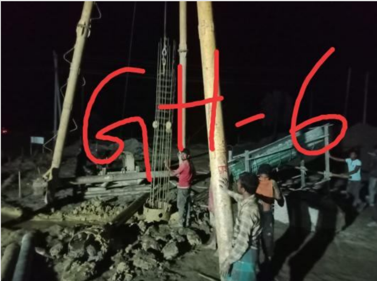
Guard House pile concreting by RMC on 19-03-23
