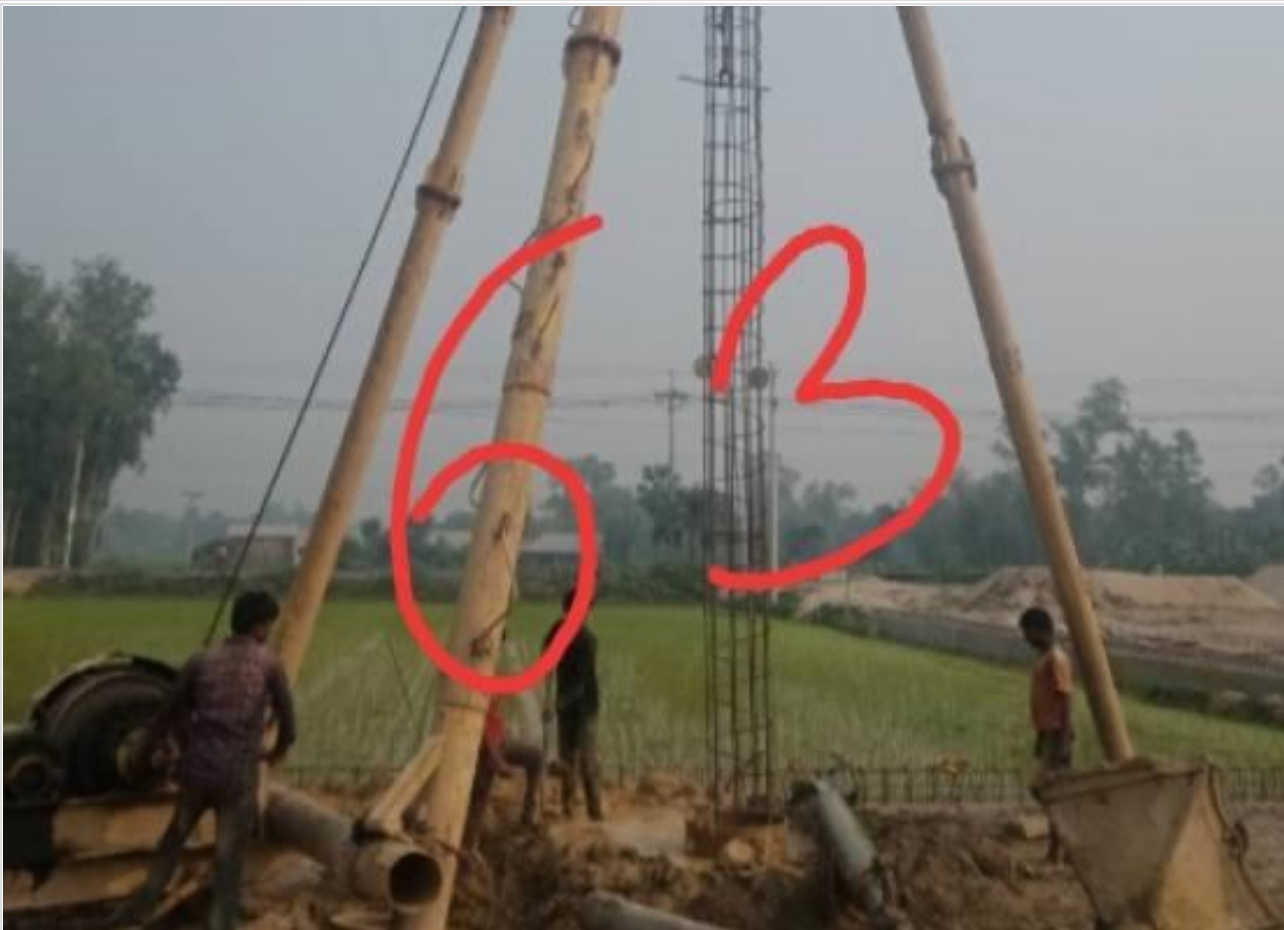
Com. Bldg. 63 Pile Boring on 14-03-23
