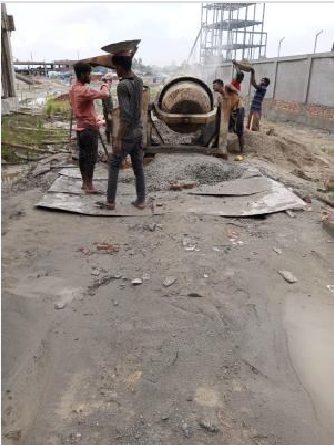
Dormitory column casting on 25-08-23
