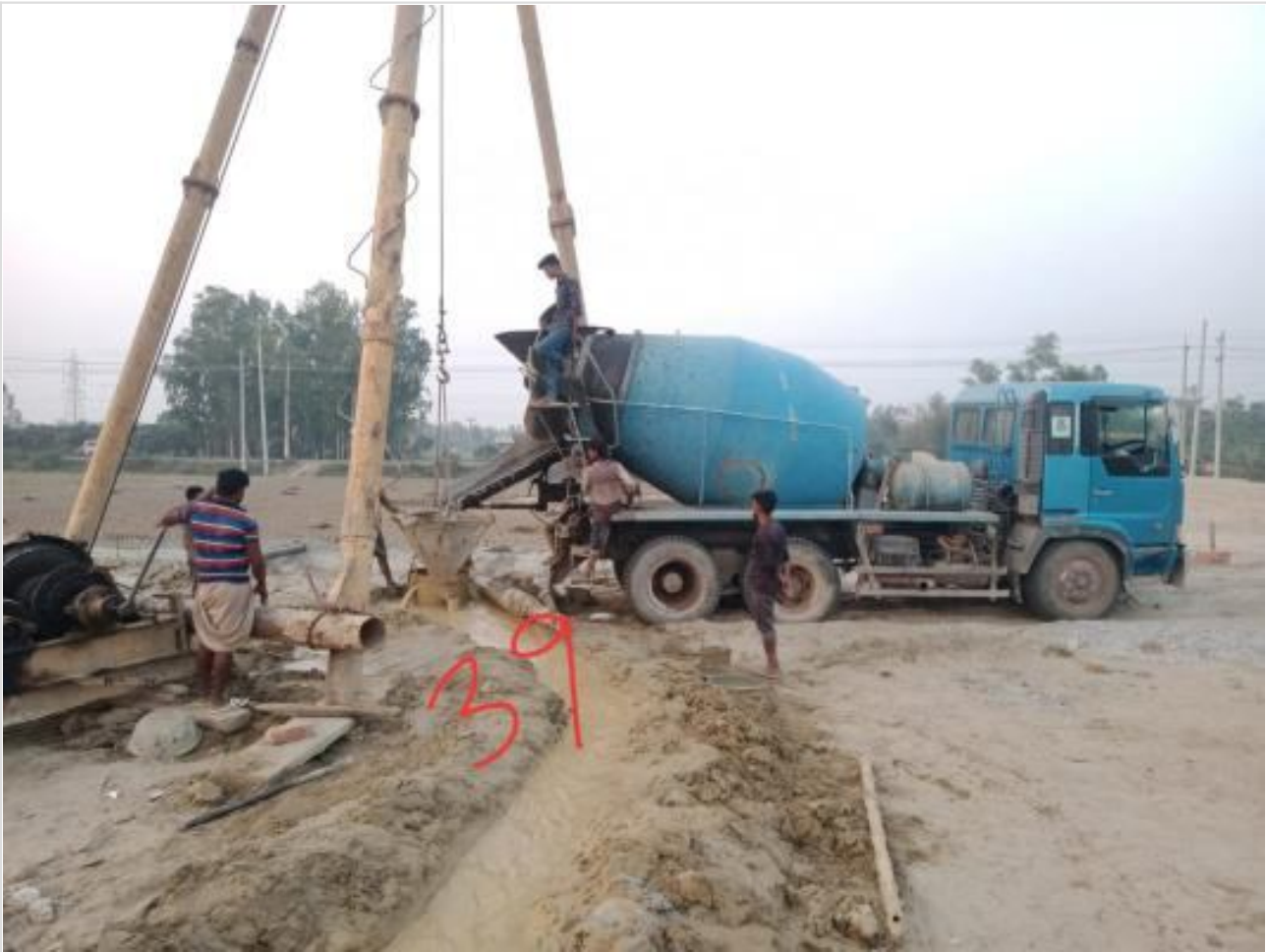
Ready mix concreting of pile on 02-03-23
