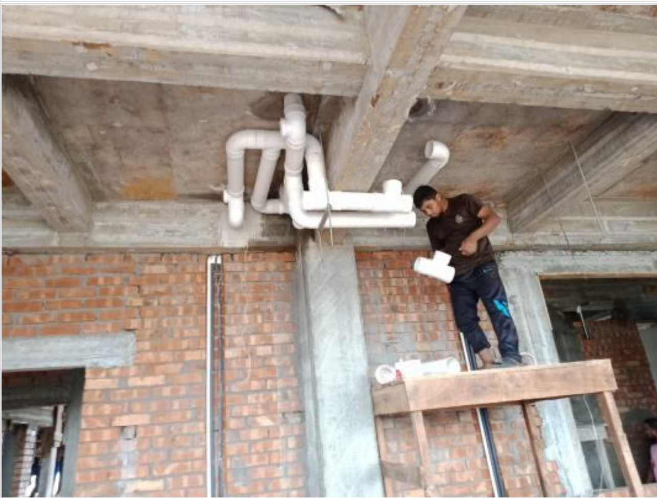
Comp. Bldg. Sanitary work on 29-08-23
