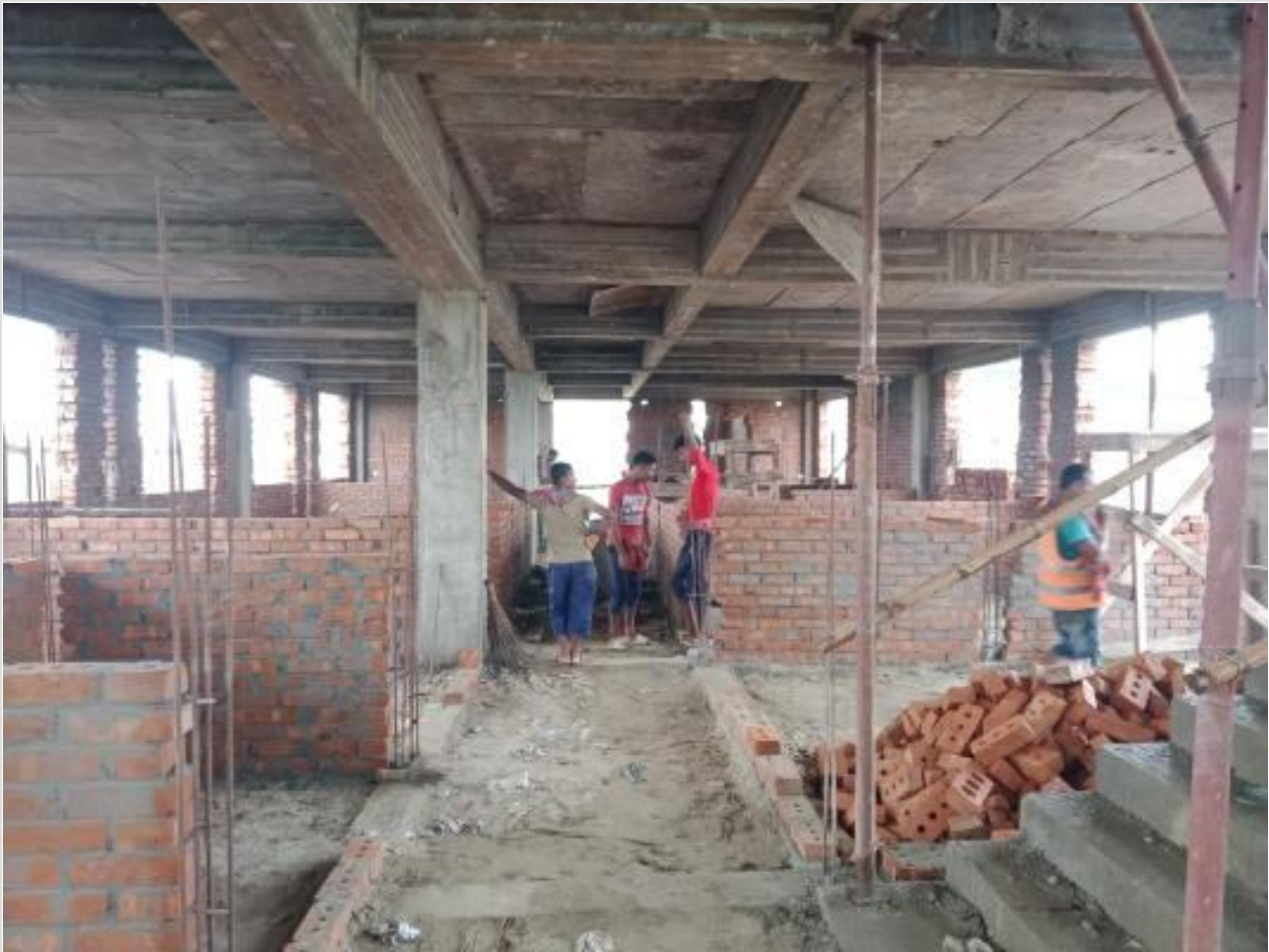
Dorm. Bldg Brick work on 25-09-23
