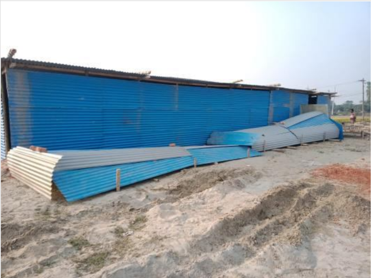
Shed completed on 22-01-23
