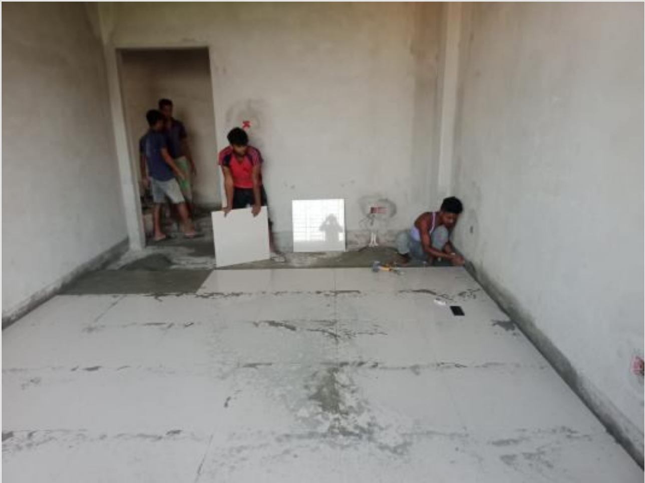
Comp. Bldg. GF Tiles work on 01-11-23
