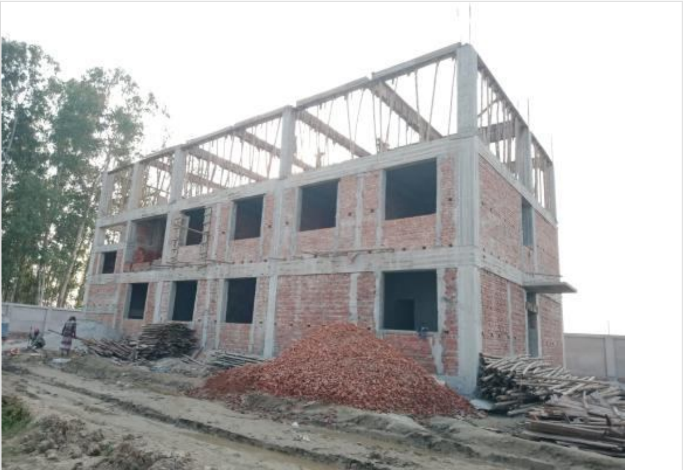
Dorm. Bldg. 2nd floor shuttering work on 06-11-23
