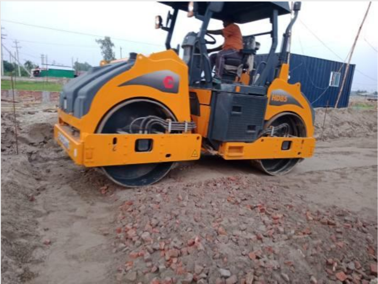
Road Sub-base work on 22-07-23
