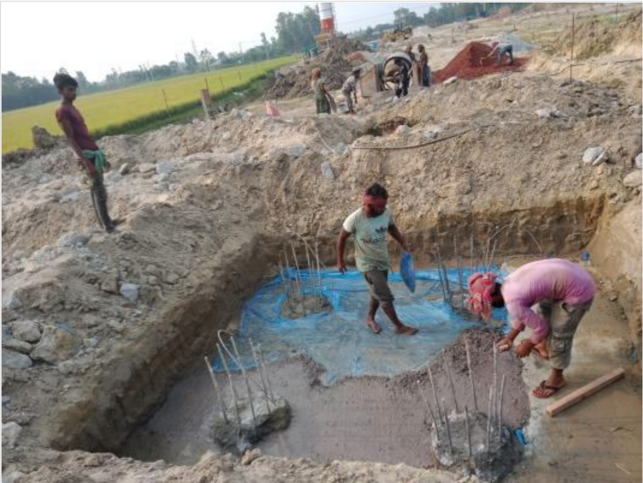
Pile cap CC work on 11-05-23
