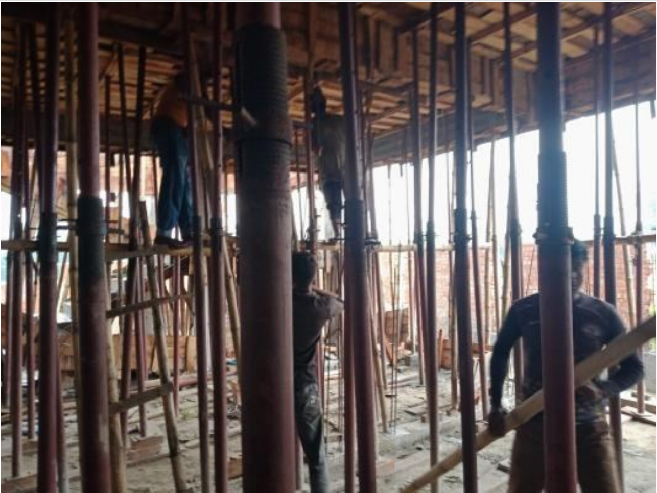
Shuttering work on 09-07-23
