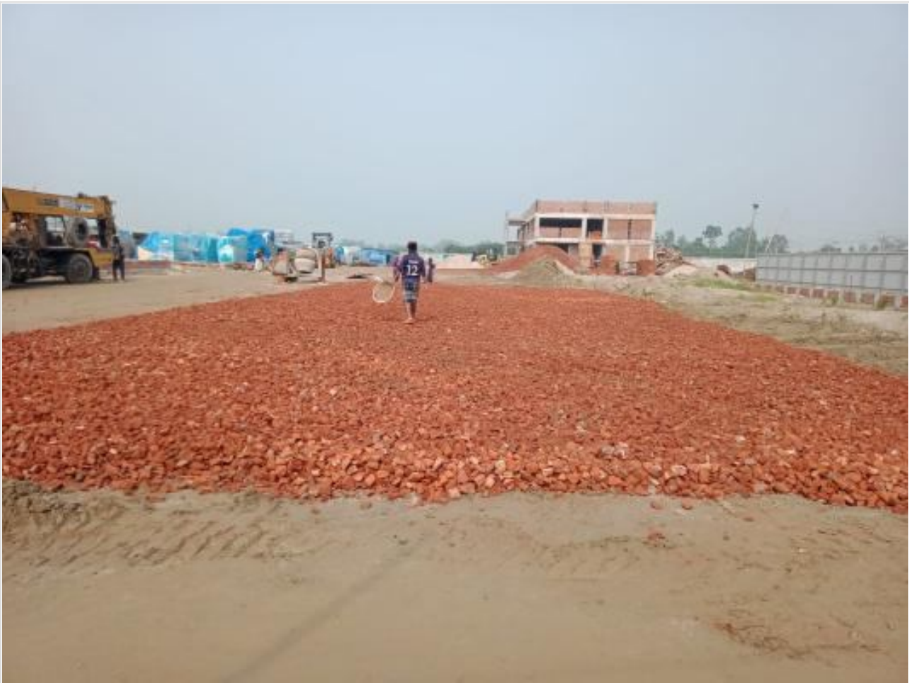
Road Sub-base work on 01-09-23
