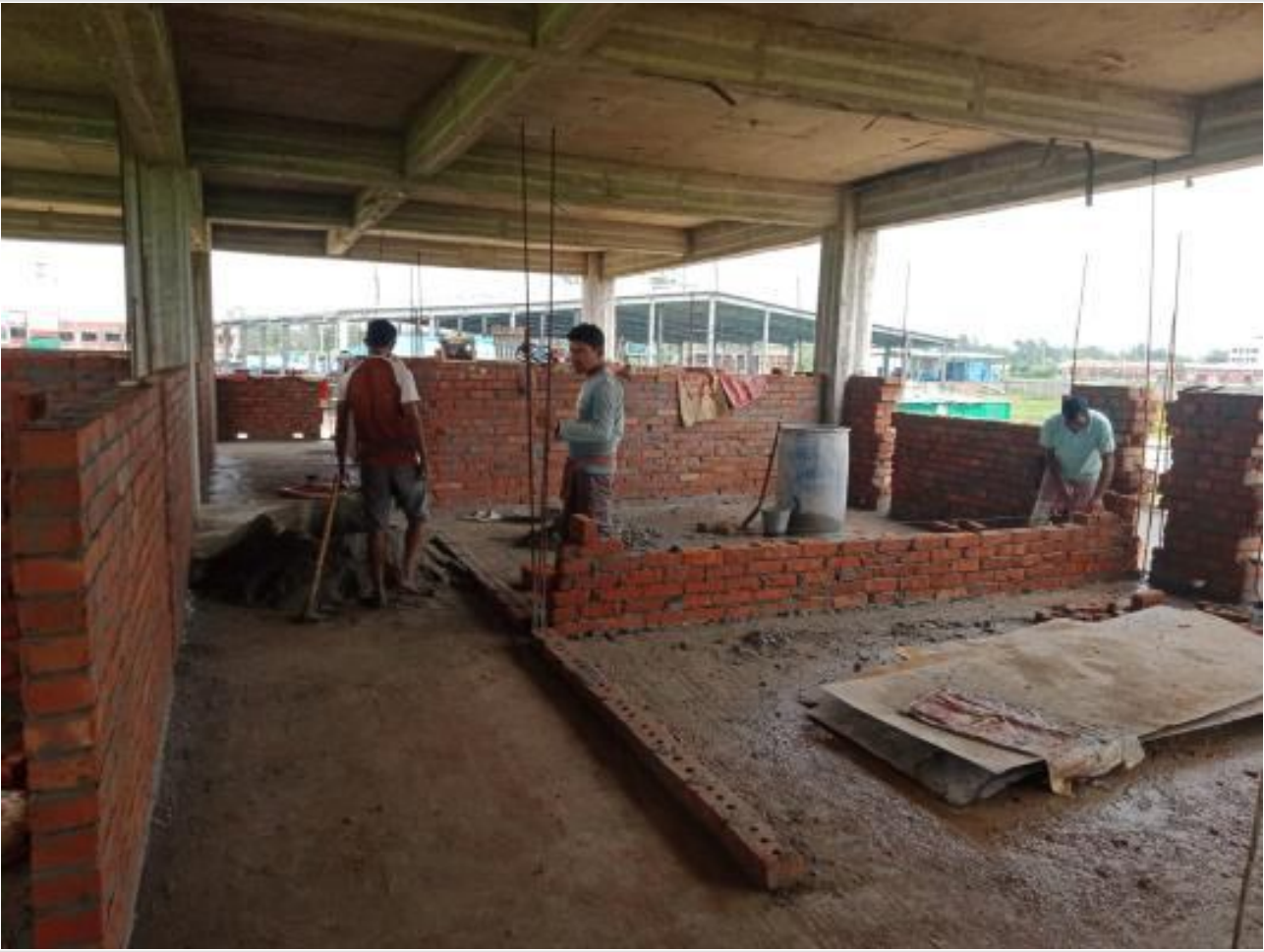
Dorm. Bldg. 1st floor brick work on 06-10-23
