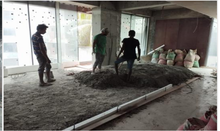
4th Flr-Floor Raising Concreting on 09-07-24
