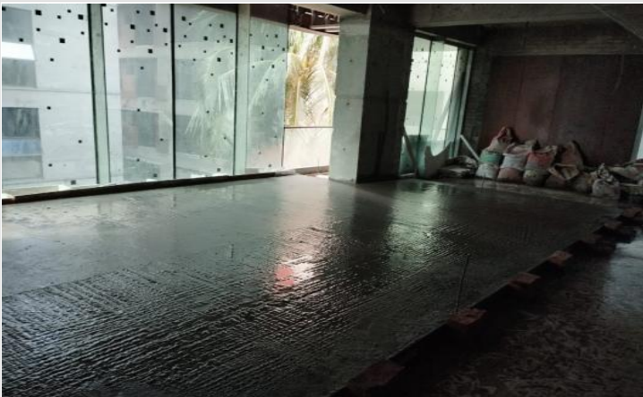
4th Flr-Floor Raising Concreting Complet on 10-07-24
