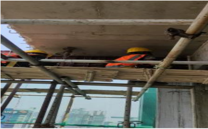
L-16-Beam Shutter removing on 29-04-23
