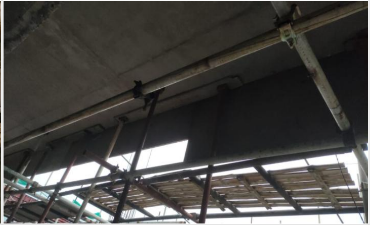
L-16-Drop Wall Shuttering on 29-04-23
