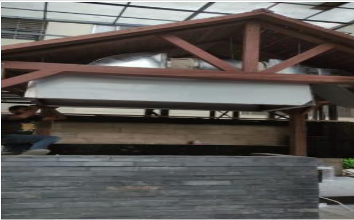
Coffee shop outside BBQ shed on 18-03-23
