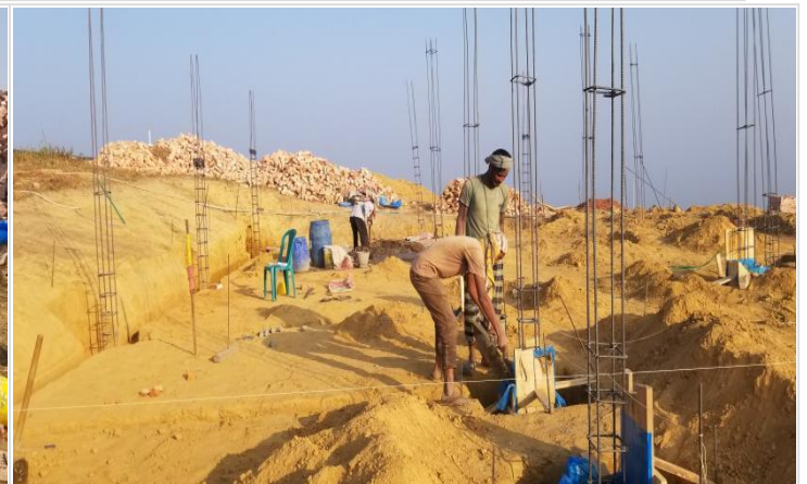
Short column casting work for guest house on 17-01-21
