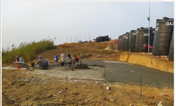
Soling joint fillup & plaster work at w on 21-01-21
