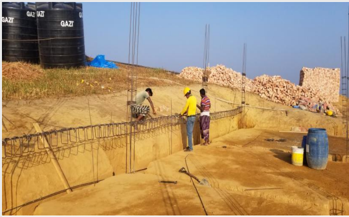
MS rod cutting & binding work for grade on 19-01-21
