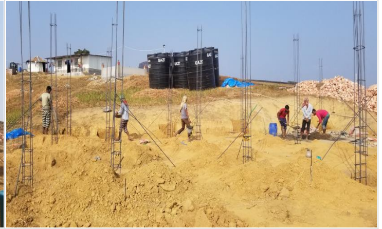
Footing casting work on going at G.House on 15-01-21
