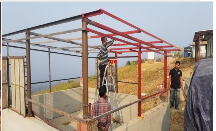
Mechanics Shed Frame Work on 20-01-21
