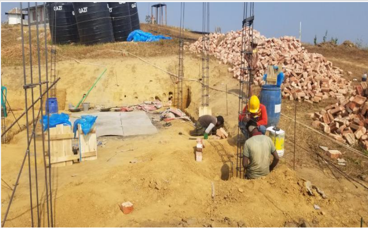
Shuttering fitting work for short column on 16-01-21
