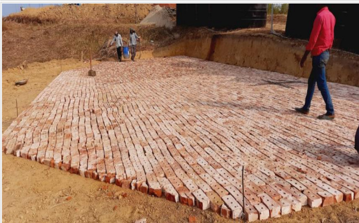
Soling for PVC Water Tank on 20-01-21
