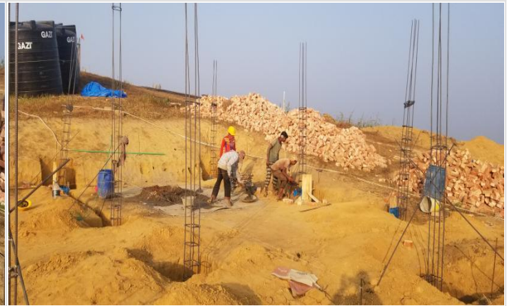
Short column casting work for guest house on 16-01-21
