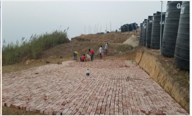
Brick soling work for water tank place on 19-01-21
