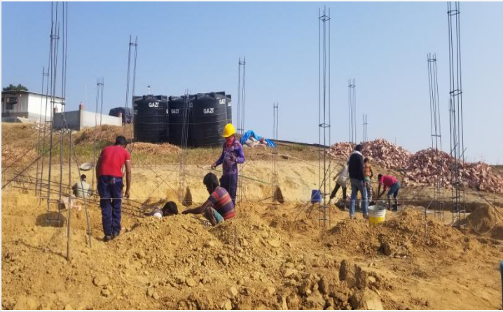
Column standing work on going at G.House on 15-01-21
