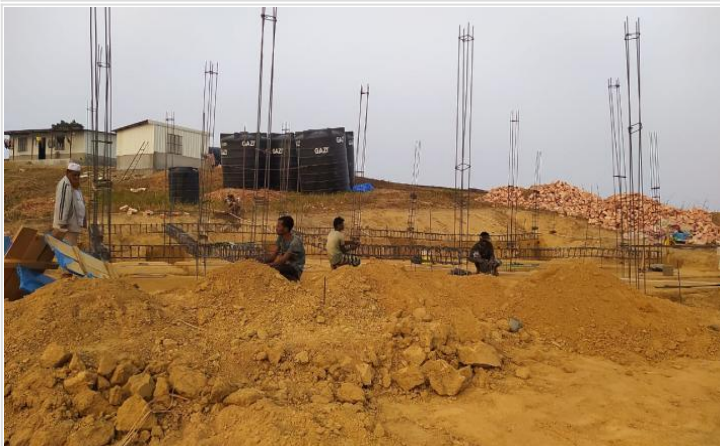
Rod binding work for grade beam at guest on 21-01-21
