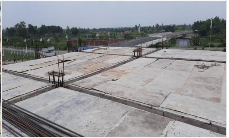
1st floor Slab Shuttering on 09-06-21
