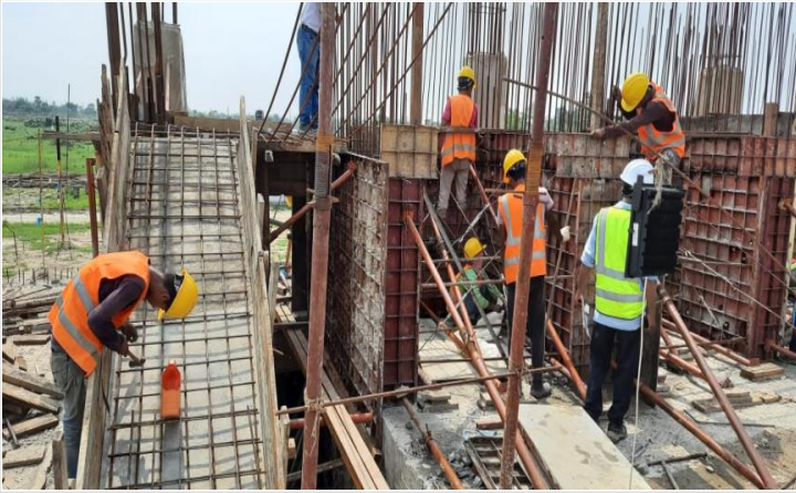
Ground Floor Stair Re-bar work on 09-06-21
