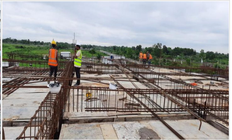
1st floor Slab Shuttering on 12-06-21
