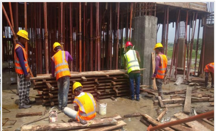
1st floor Slab Shuttering on 15-06-21
