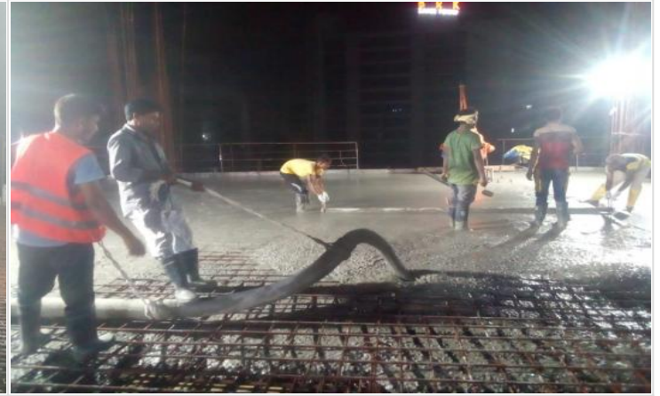
South Tower 11th Floor Slab Concreting on 02-09-21
