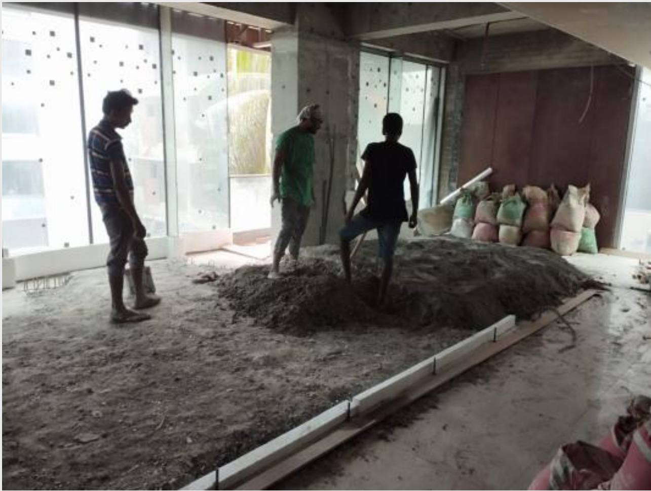
4th Flr-Floor Raising Concreting on 09-07-24
