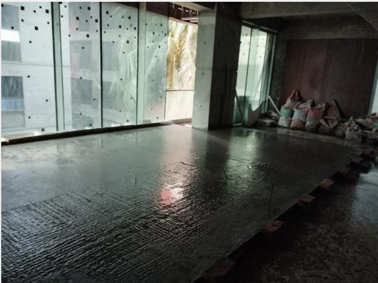
4th Flr-Floor Raising Concreting Complet on 10-07-24
