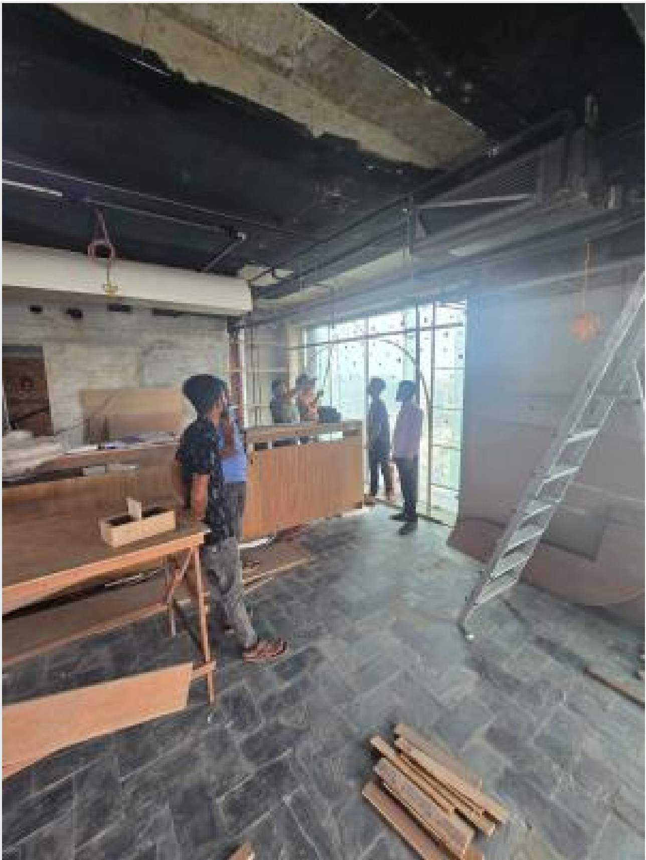
14th Floor Interior Works on 09-07-24
