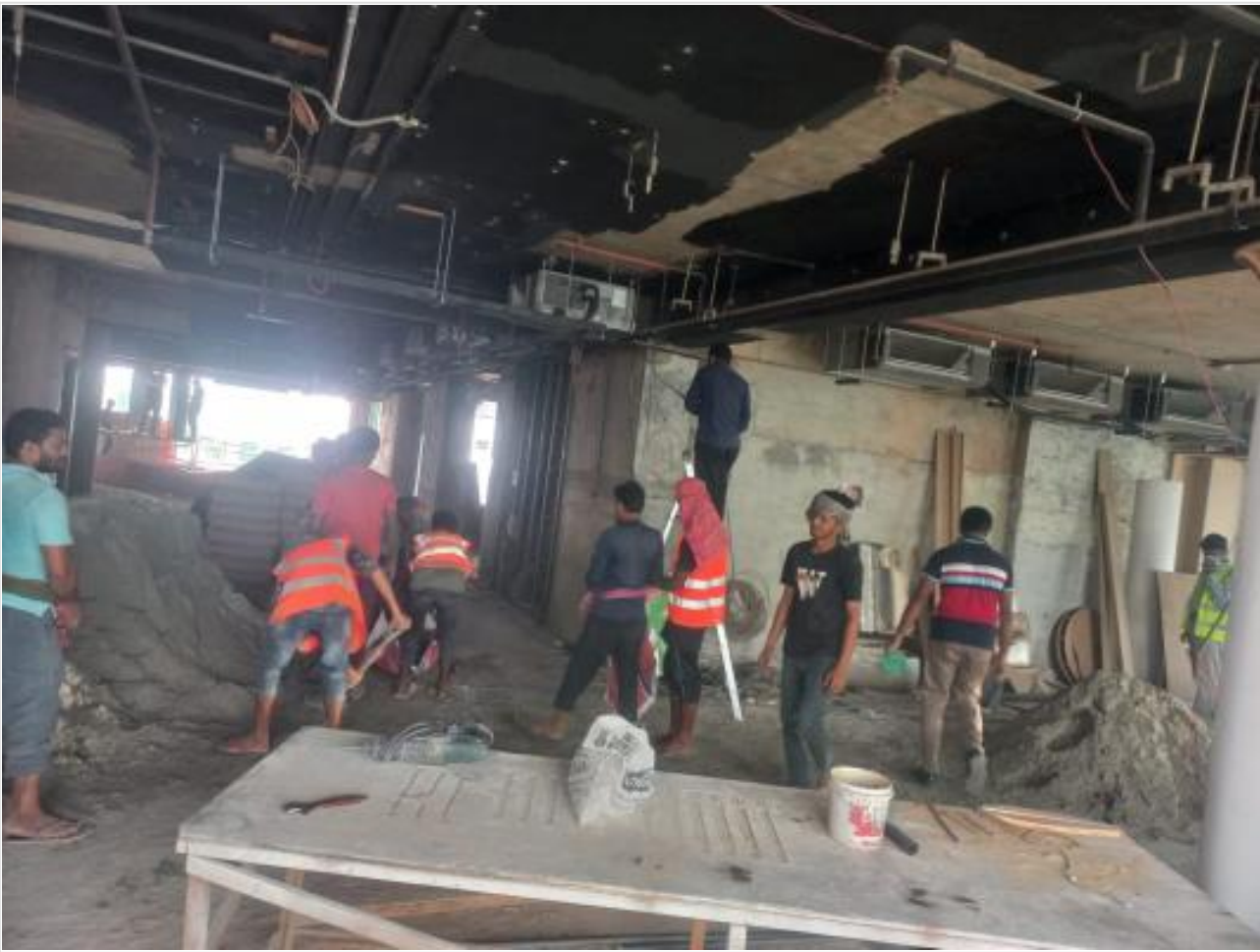
L-16-Materials Removal on 29-11-23
