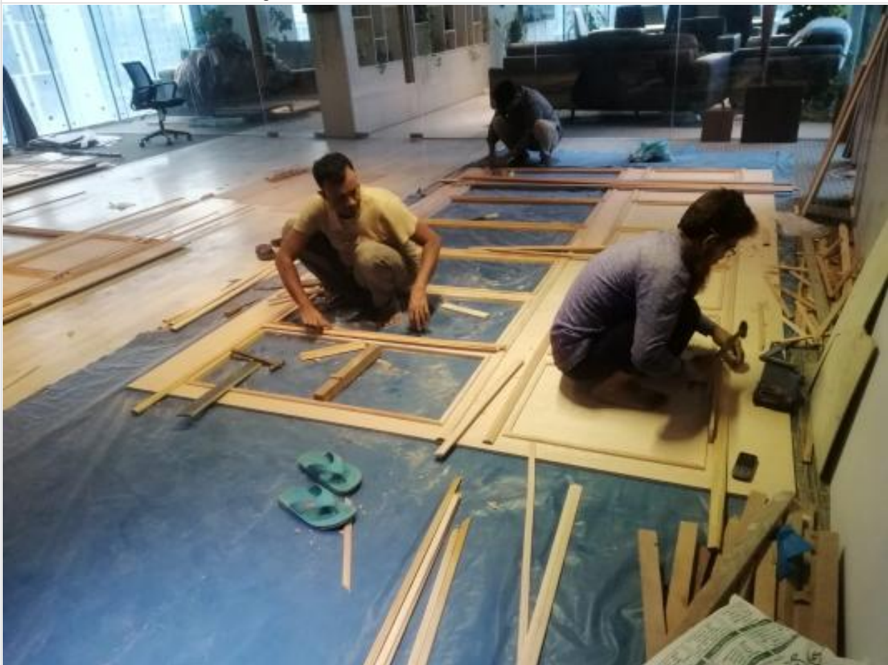
L-11-Lounge Outside Glass Frame on 28-12-23
