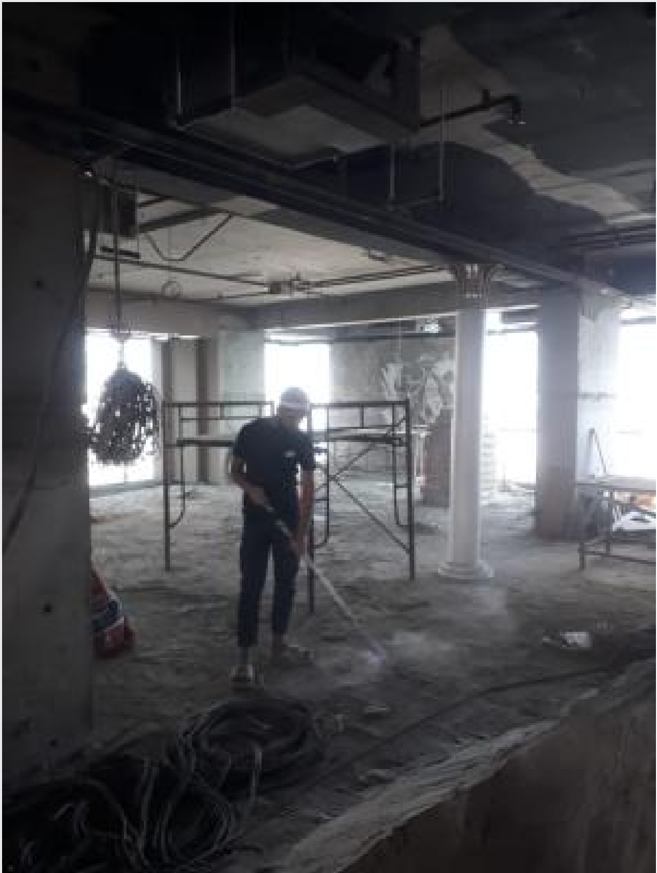
L-16-Materials Removal on 25-11-23
