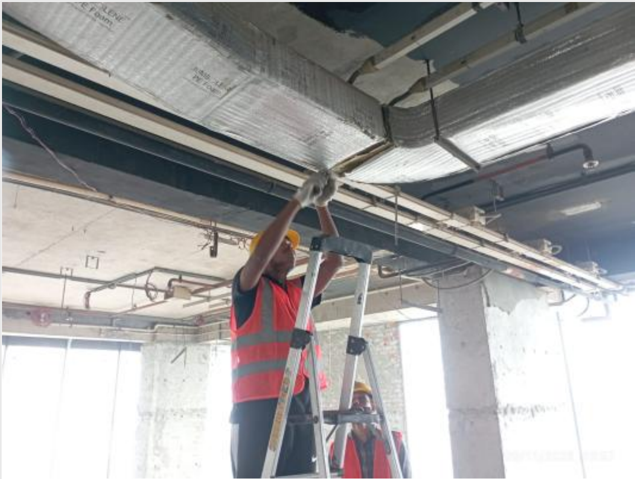
L-14-Old AC duct removing on 09-11-23
