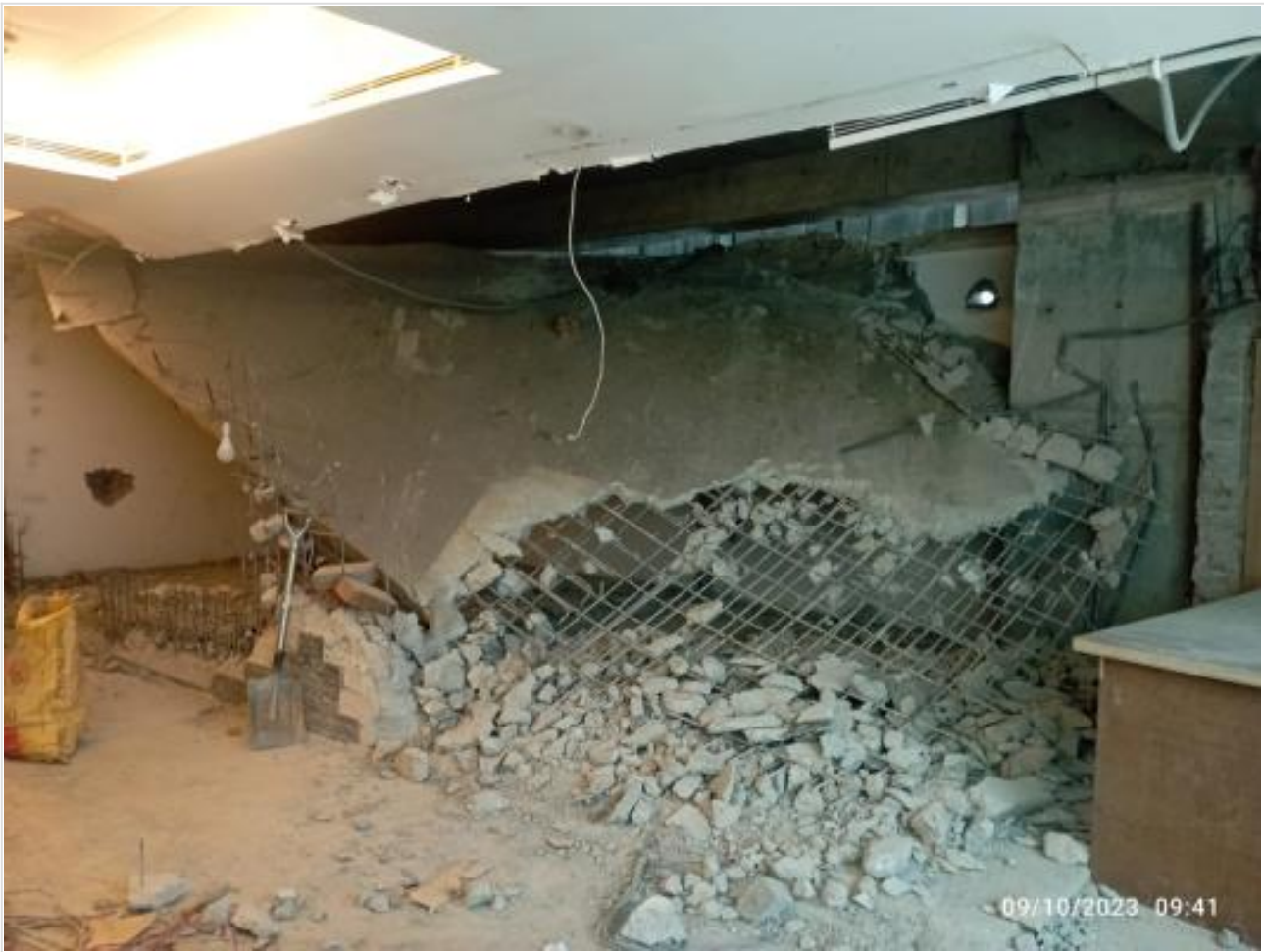
L-4-North-East Vault dismantling on 08-10-23
