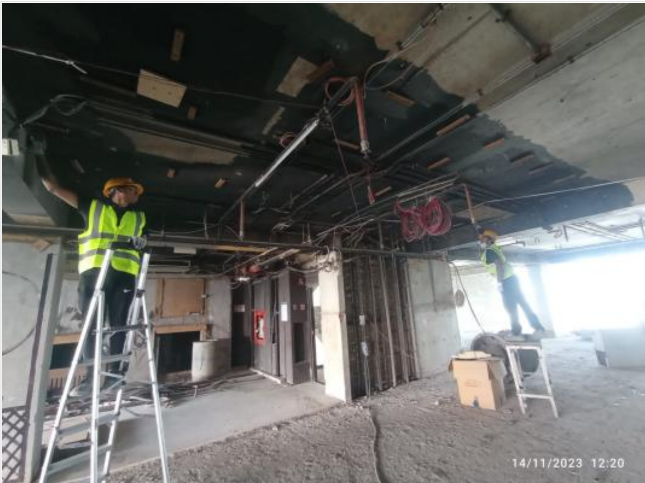
L-14-AC installation on 14-11-23
