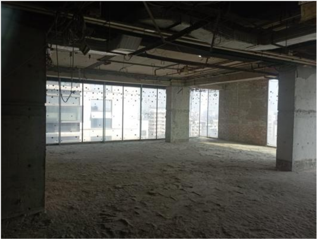
L-14-Old Kitchen Area on 25-10-23
