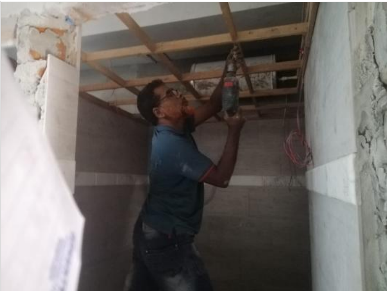
L-11-Steam-Suana-False Ceiling on 28-12-23
