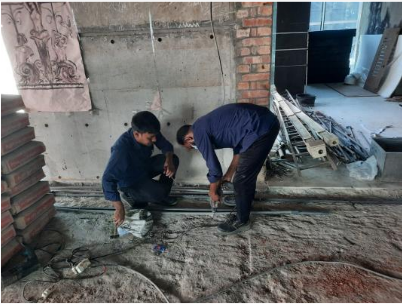
L-14-Electrical Pipe laying on 28-11-23
