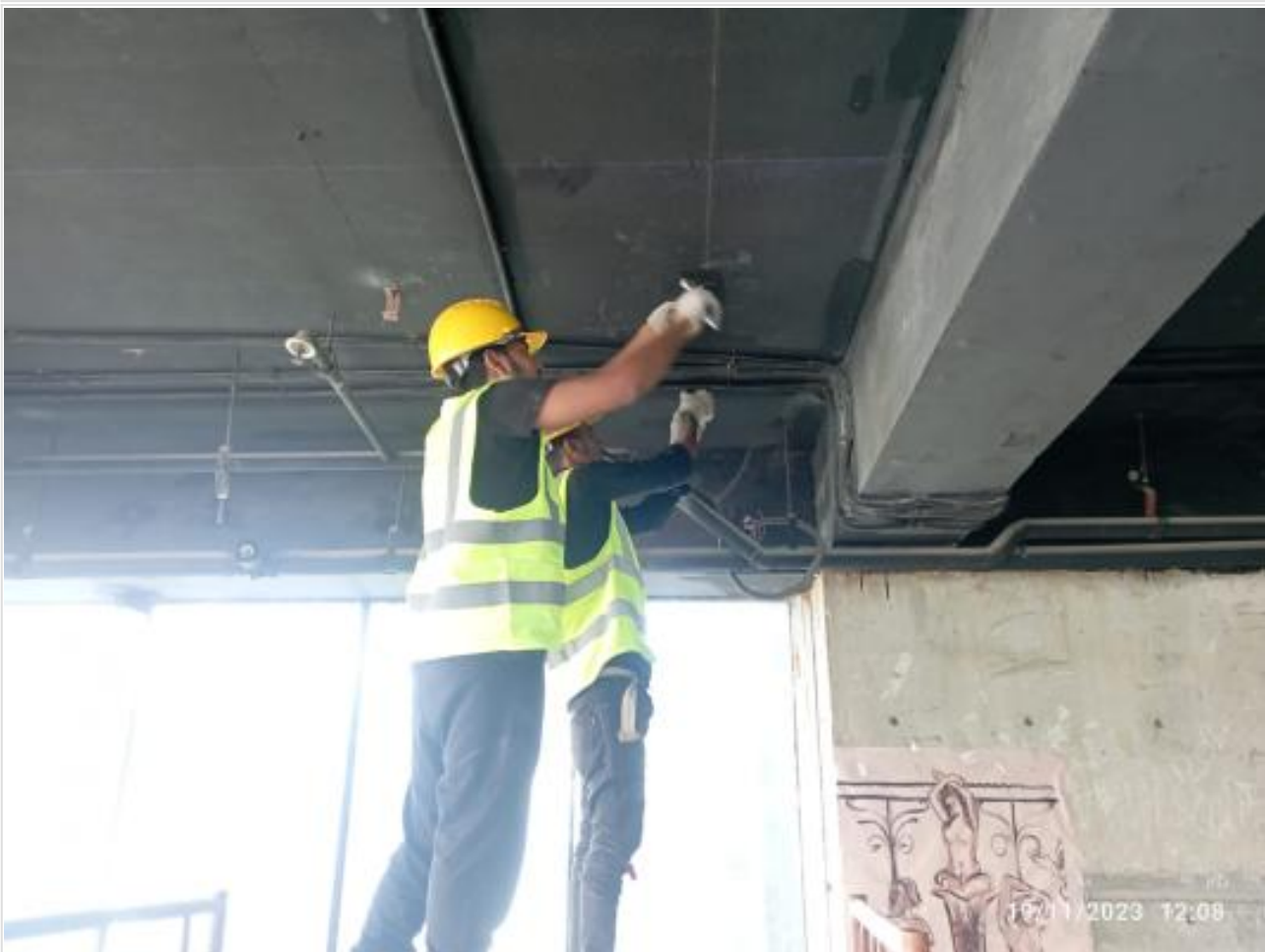
L-14-AC Installation on 19-11-23
