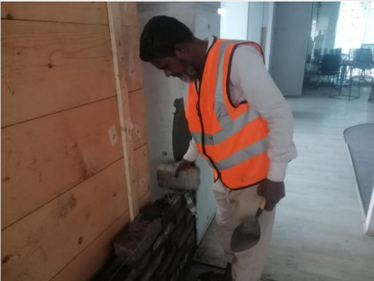
L-11-Steam n Suana-Brickwork on 29-11-23
