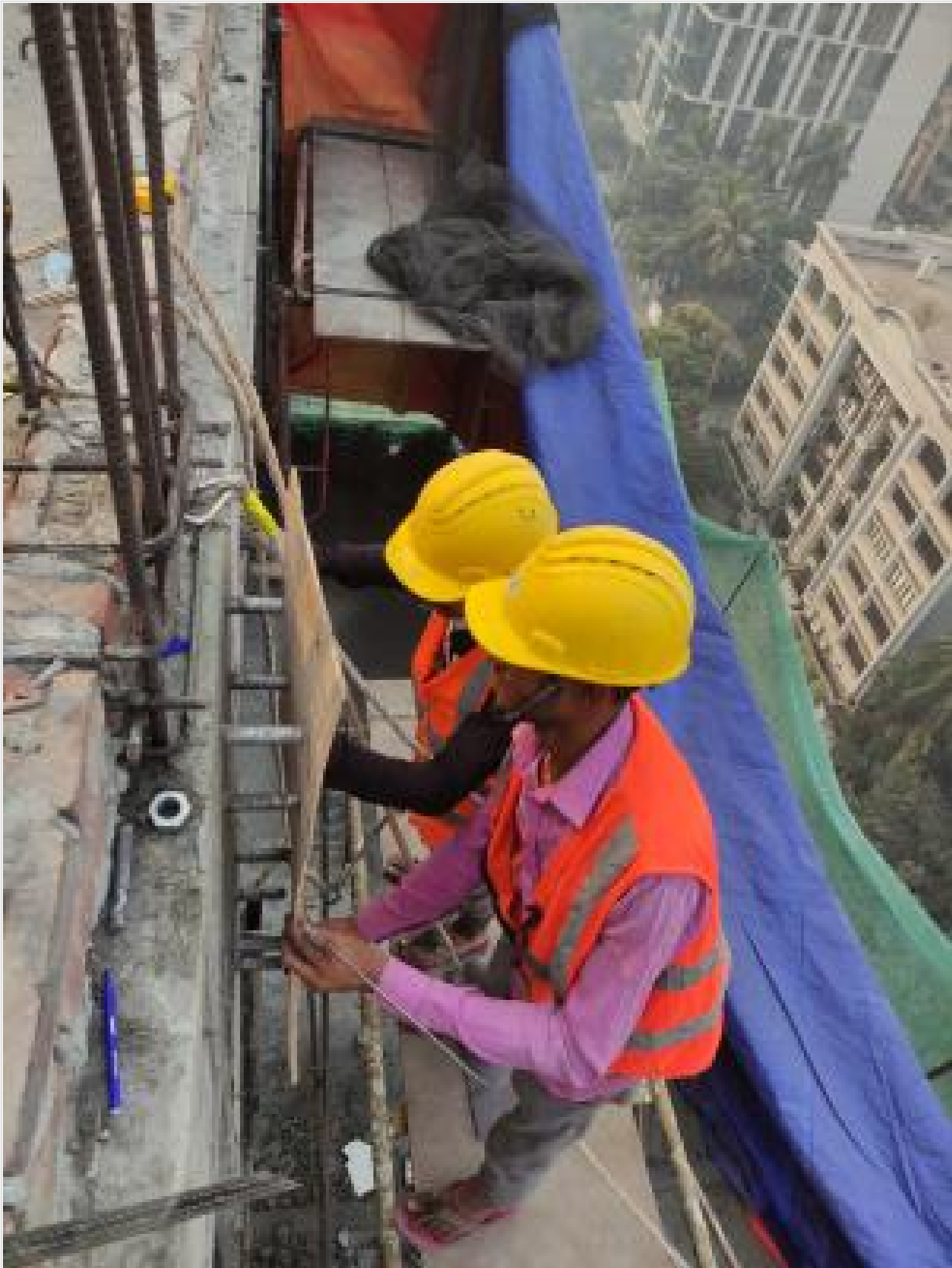
L-15-Steel Fabrication on 18-02-23
