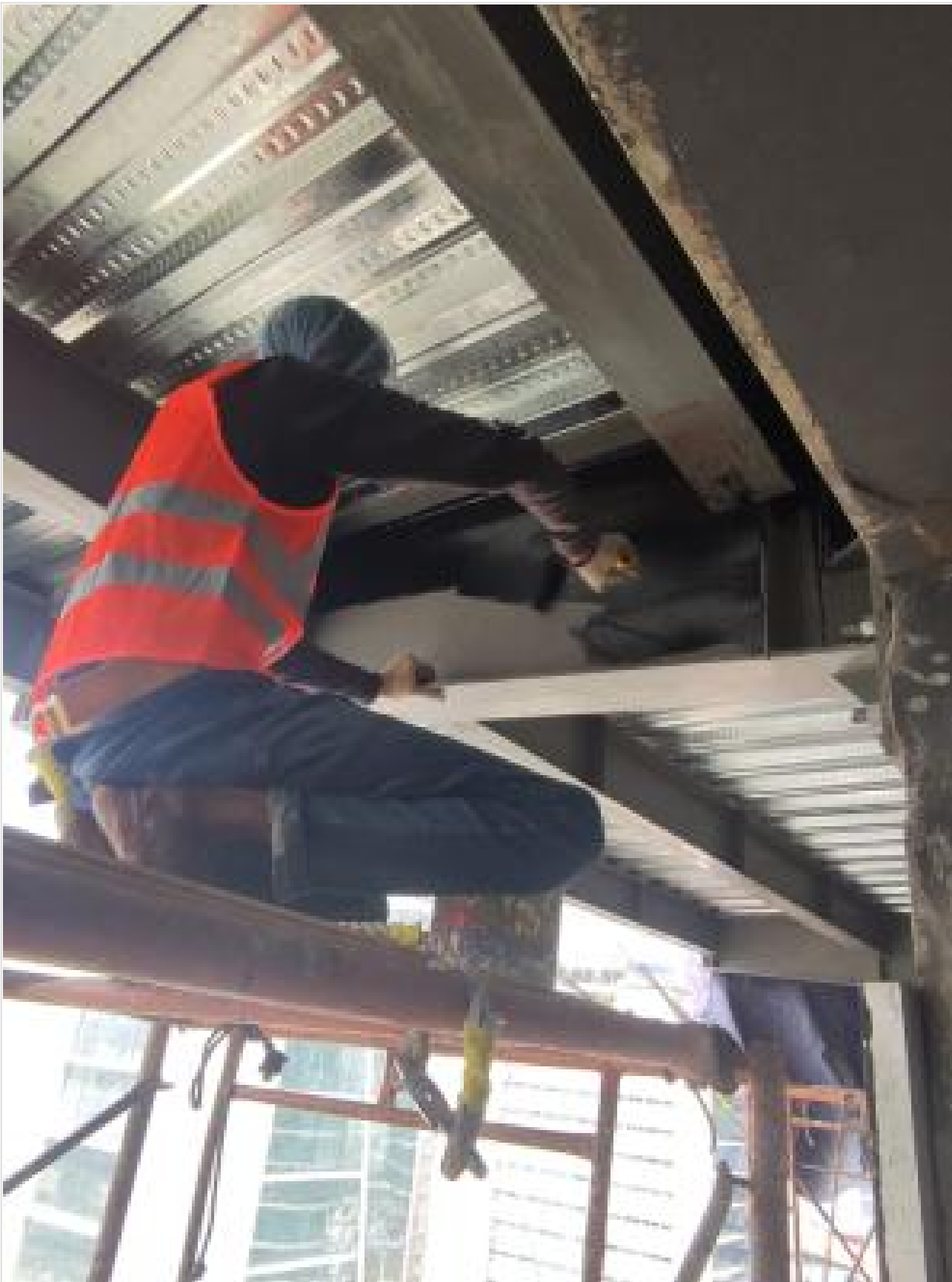
L-14-Ext Decking and Beam Painting on 27-02-23
