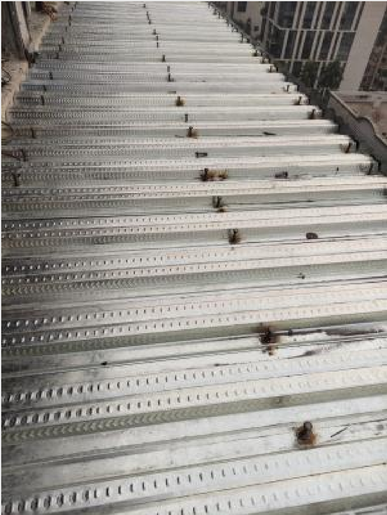
Level-14 Decking Slab complete on 13-02-23
