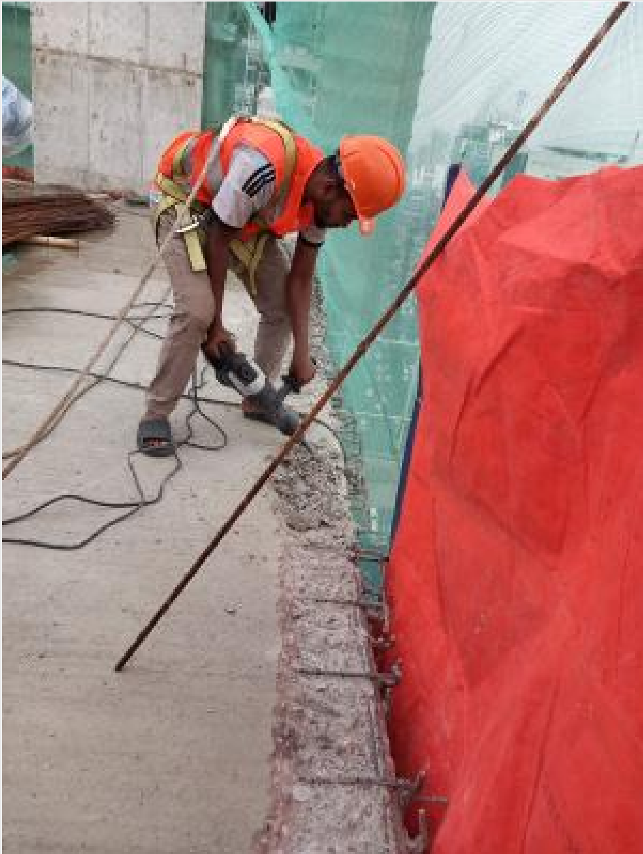
L-16-Dropwall old concrete dismantling on 29-03-23
