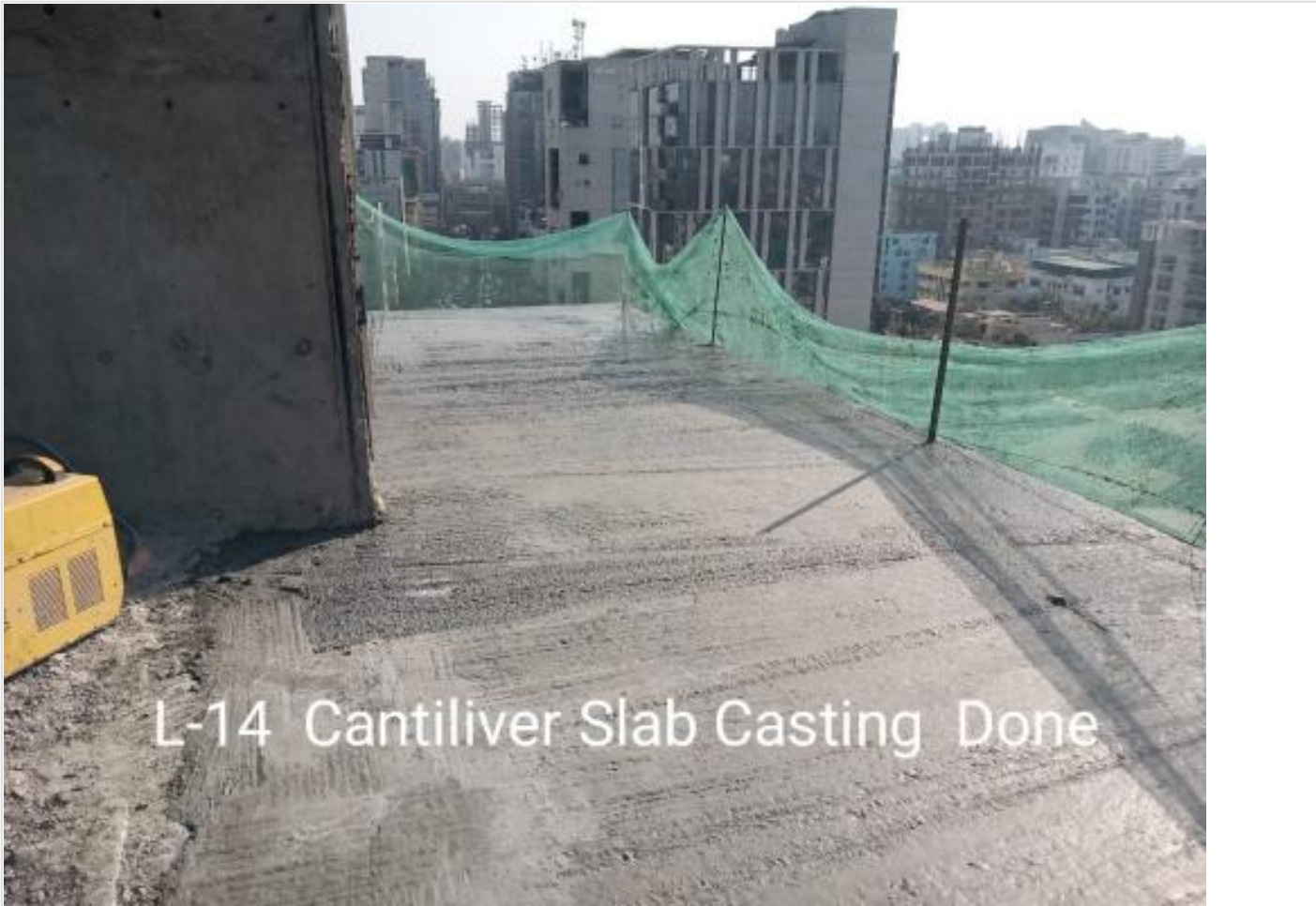
Level-14 Slab concrete completed on 13-02-23
