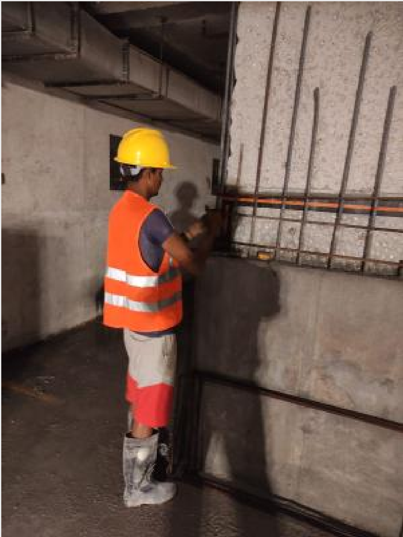
B-2 Col retrofit re-bar work on 20-02-23
