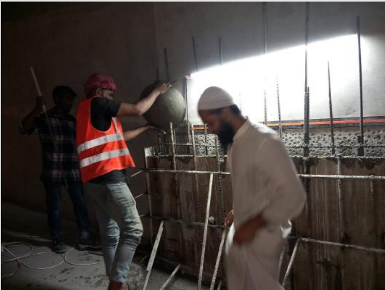
B-2-Column retrofit concreting on 29-03-23
