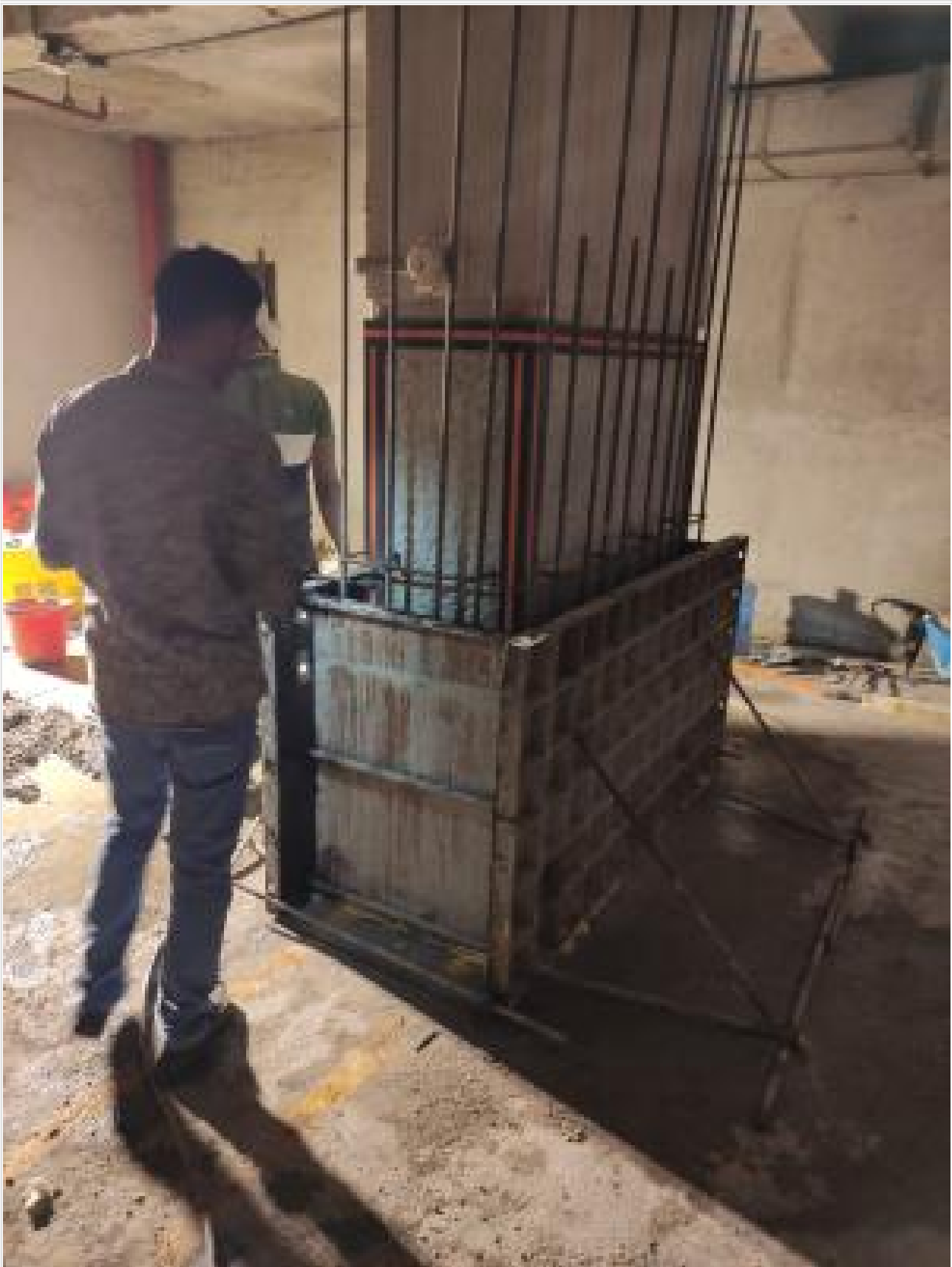
Basement-2-Column retrofitting on 08-02-23
