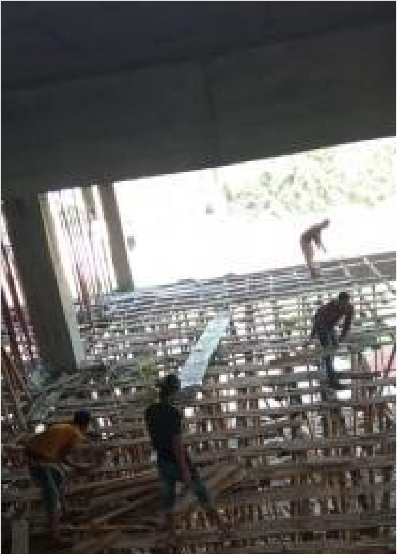
Roof Slab Shuttering on 02-05-21
