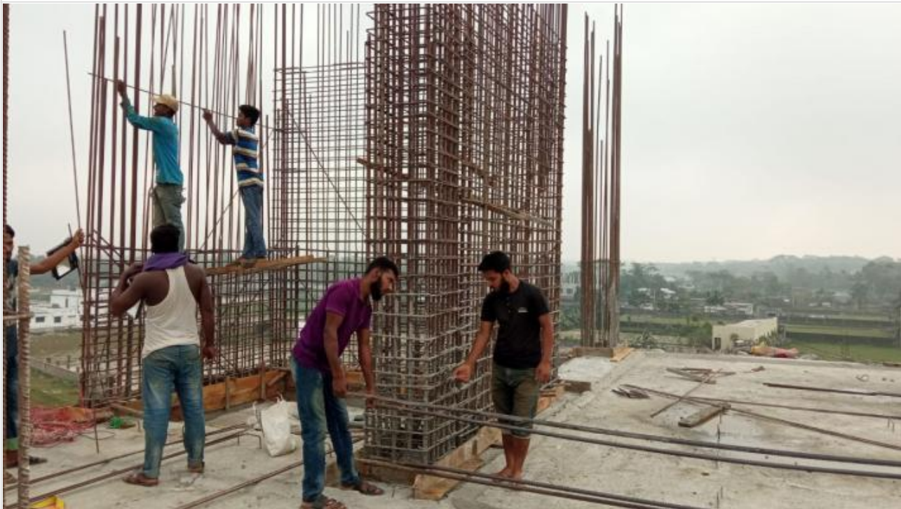
Tower-1-3rd Floor Lift Core Re-bar Work on 02-03-21
