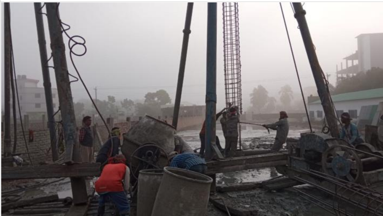
Tower-2-Pile Work on 04-12-20
