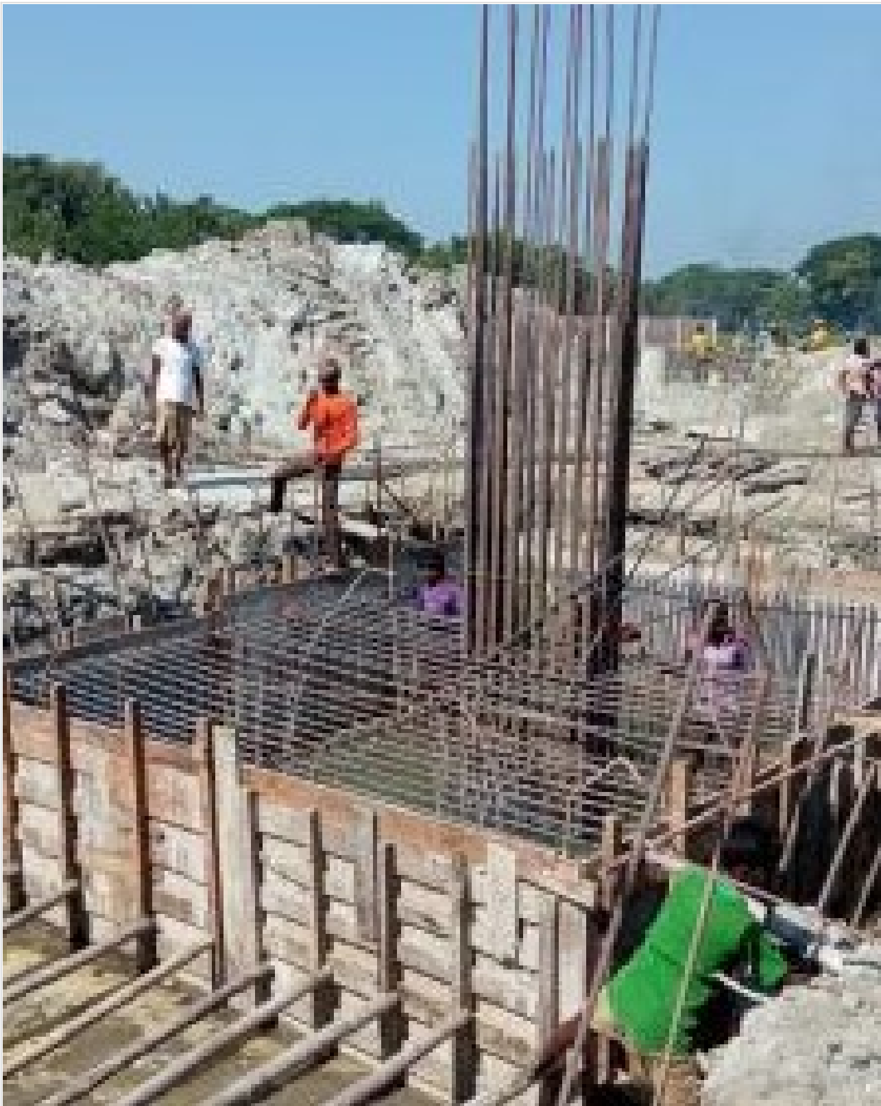
Tower-1 Pile Cap on 12-11-20
