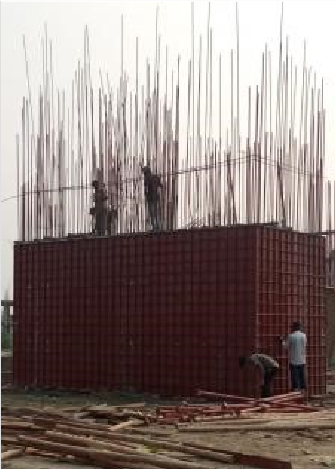
Lift Core Wall Shuttering on 24-03-21
