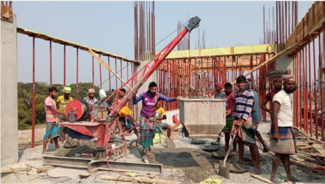
Tower-1-1st Floor Roof Slab 3600 sft Con on 07-02-21
