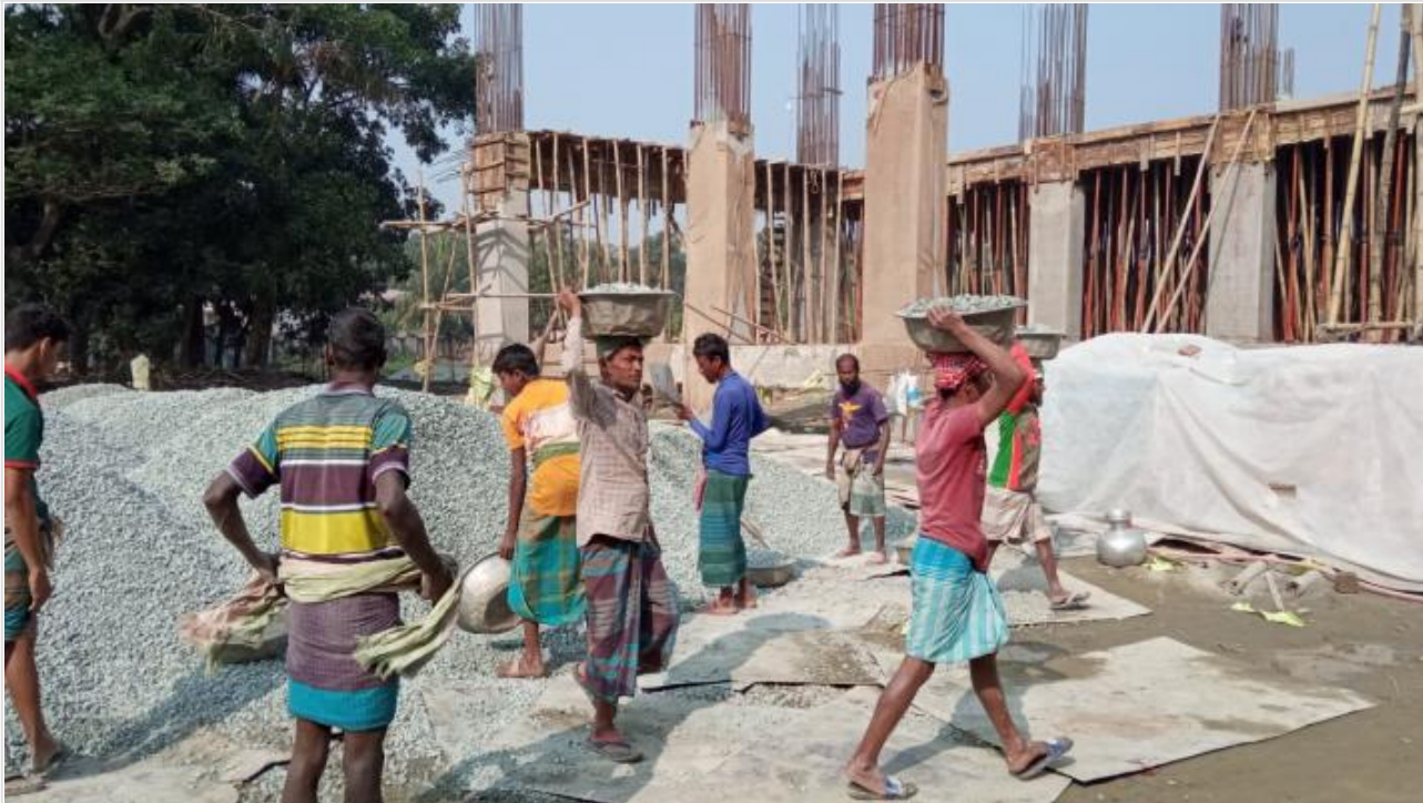
Tower-1-GF Roof Slab Concreting on 21-12-20
