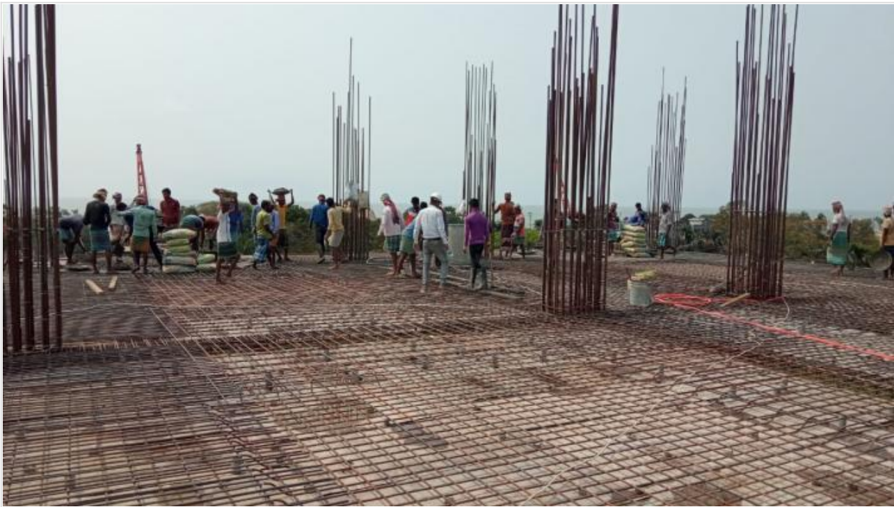
Tower-1-3rd Floor Roof Slab Concreting on 11-03-21
