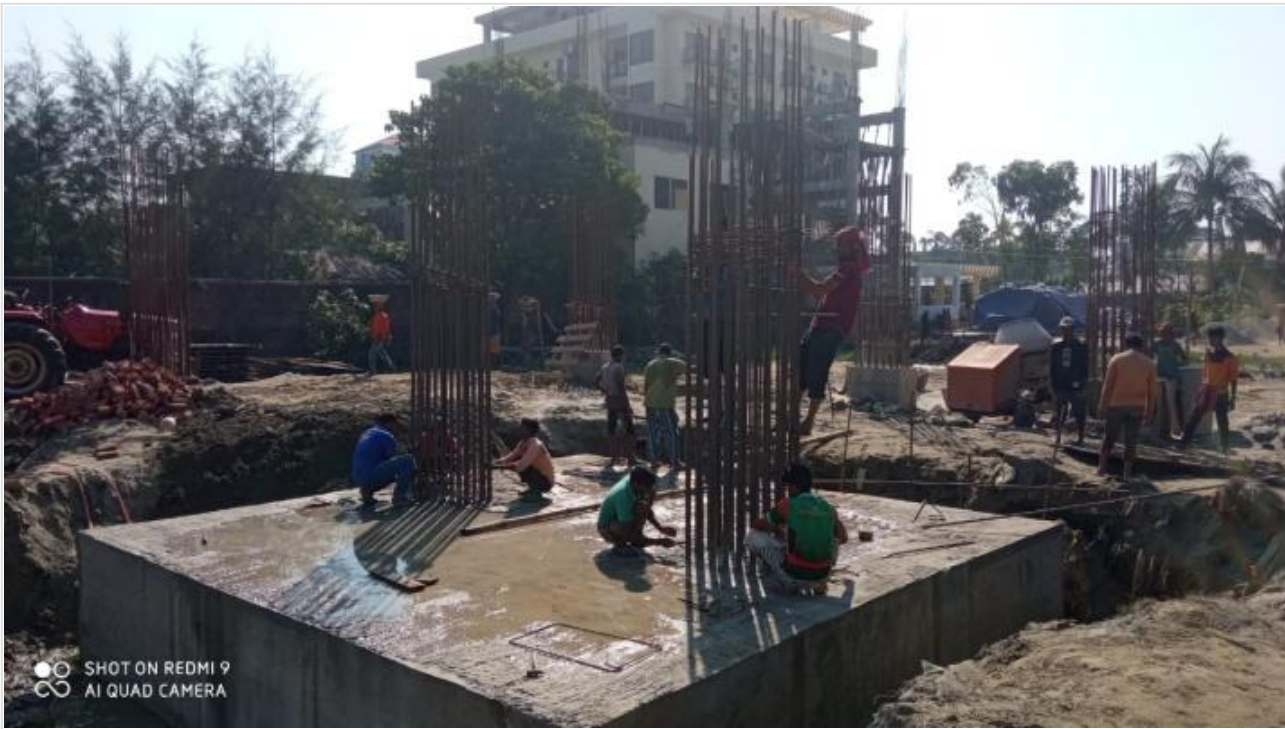
Tower-1 Pile Cap on 30-11-20
