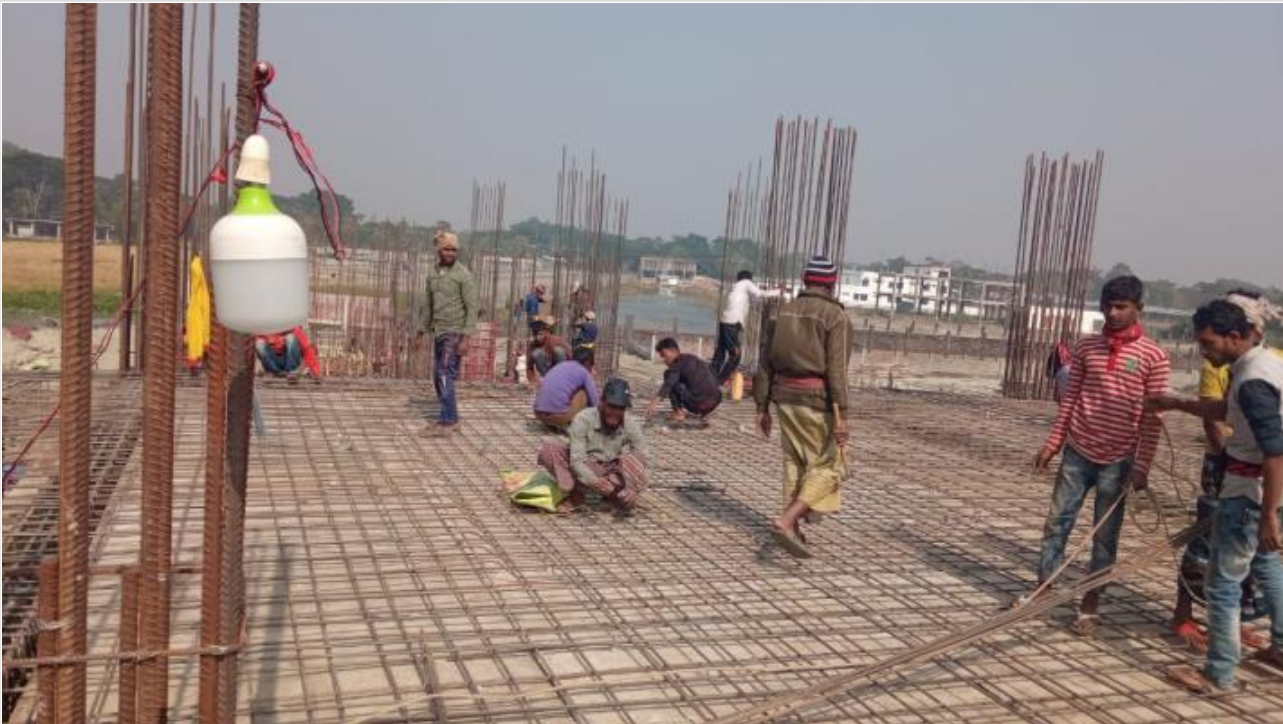
Tower-1-GF Slab Re-bar Work on 20-12-20
