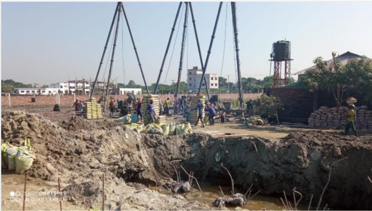
Tower-2-Piling Work on 28-11-20
