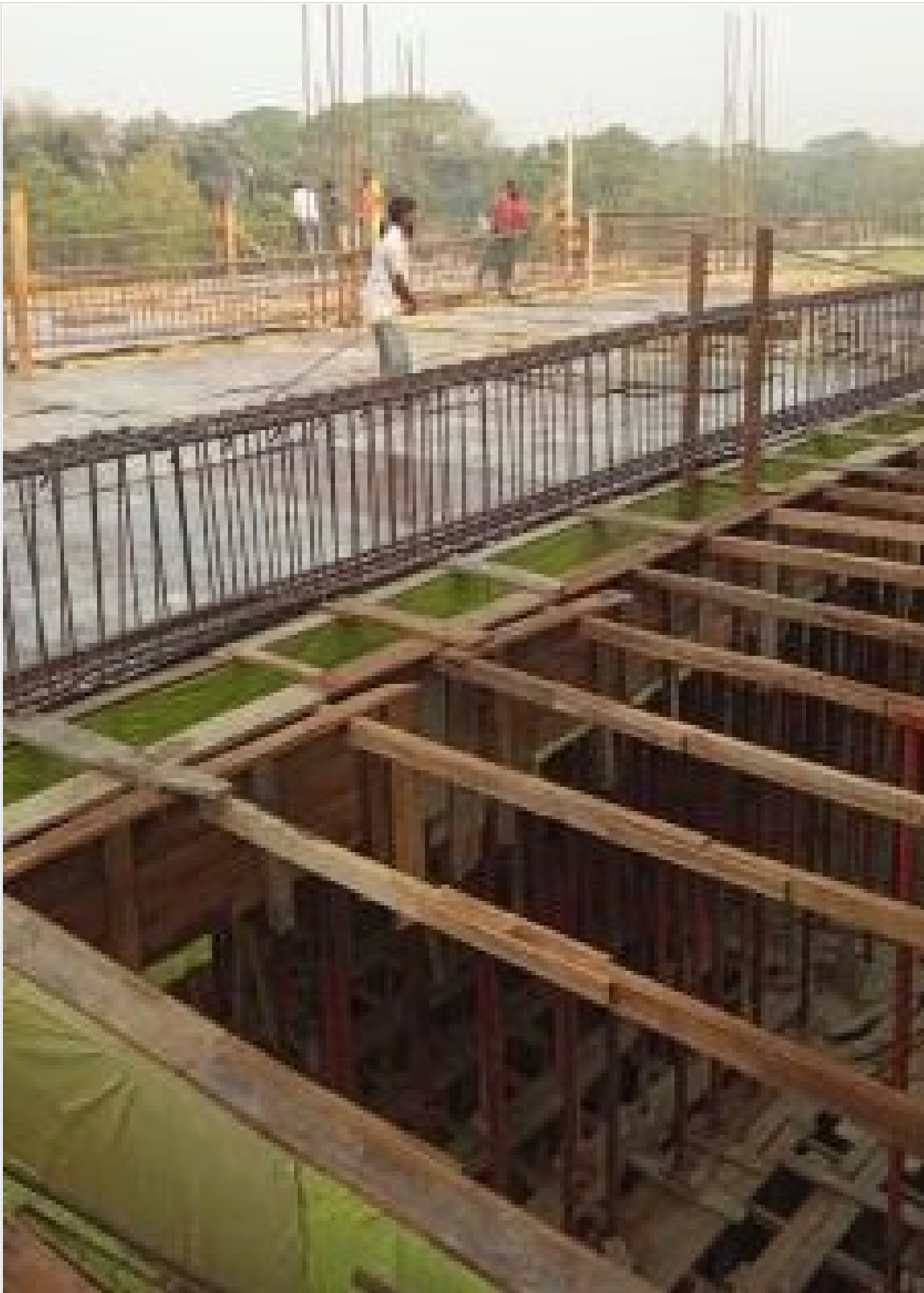
Tower-1-3rd Floor Roof Slab Shuttering on 13-03-21
