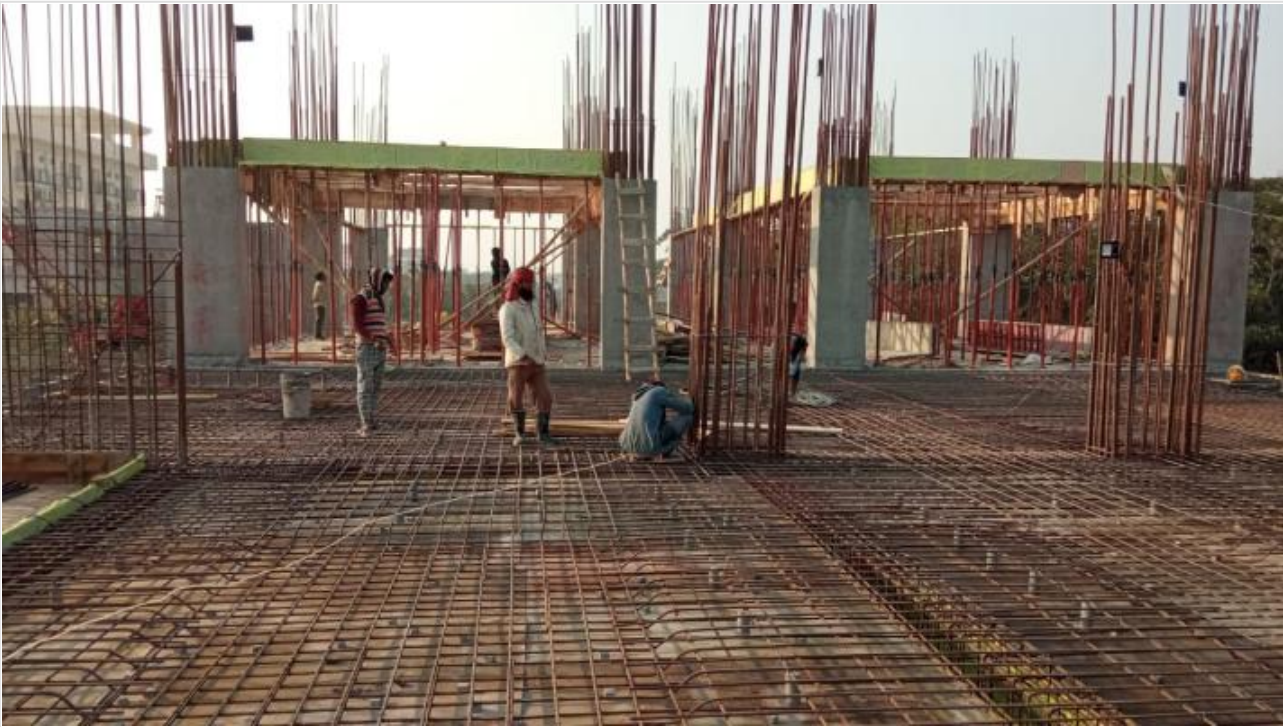
Tower-1-1st Floor Roof Slab 3600 sft Con on 05-02-21
