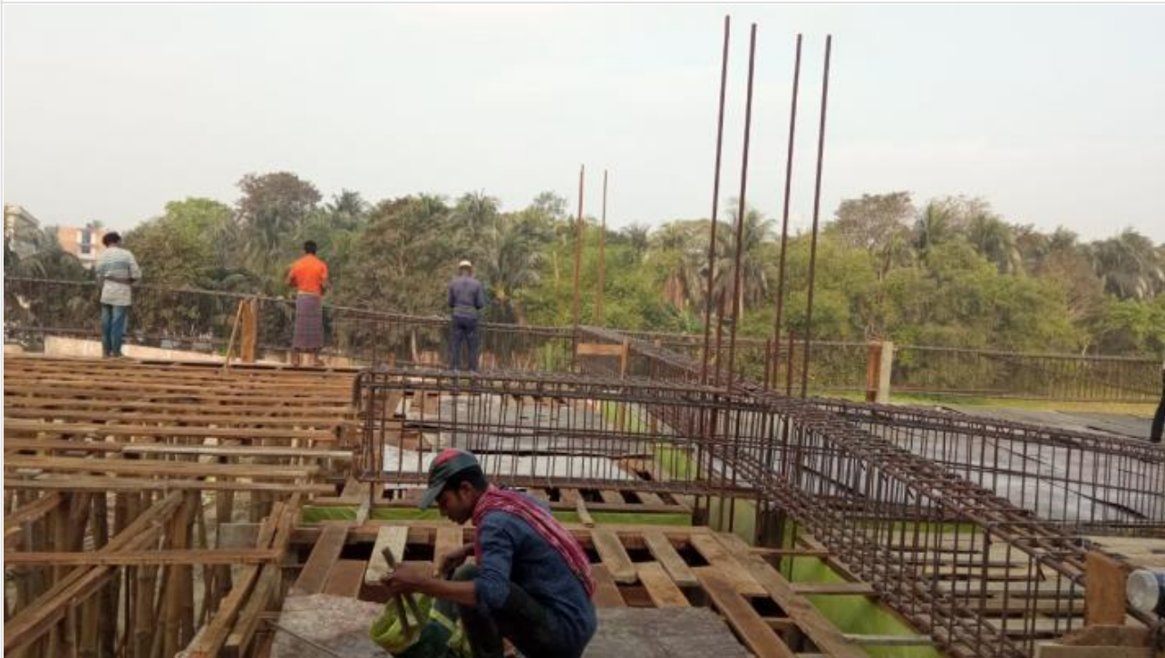
Resturant Area Slab Shuttering on 28-02-21
