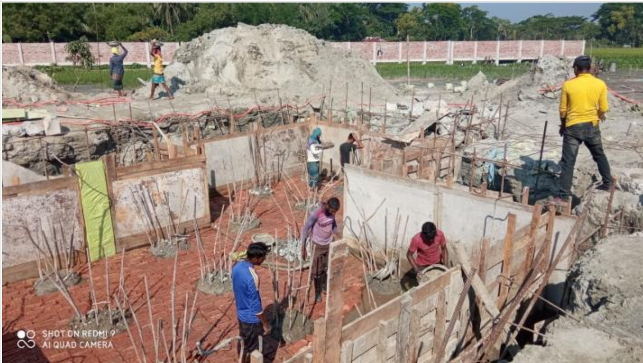
Tower-1-Pile Cap Work on 28-11-20
