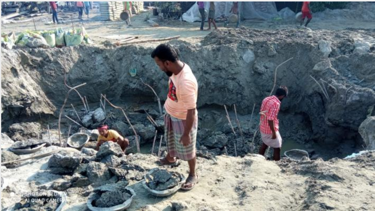
Tower-1-Pilehead breaking on 30-11-20
