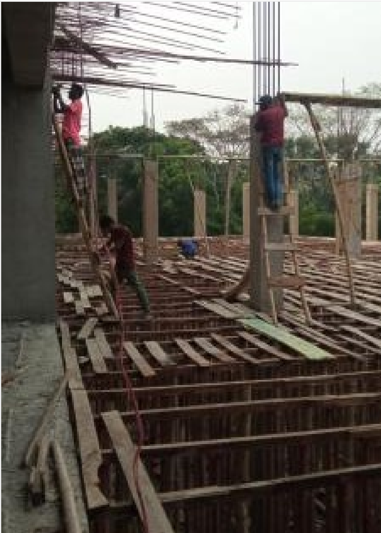
Tower-1-3rd Floor Roof Slab-Beam Shutter on 23-03-21
