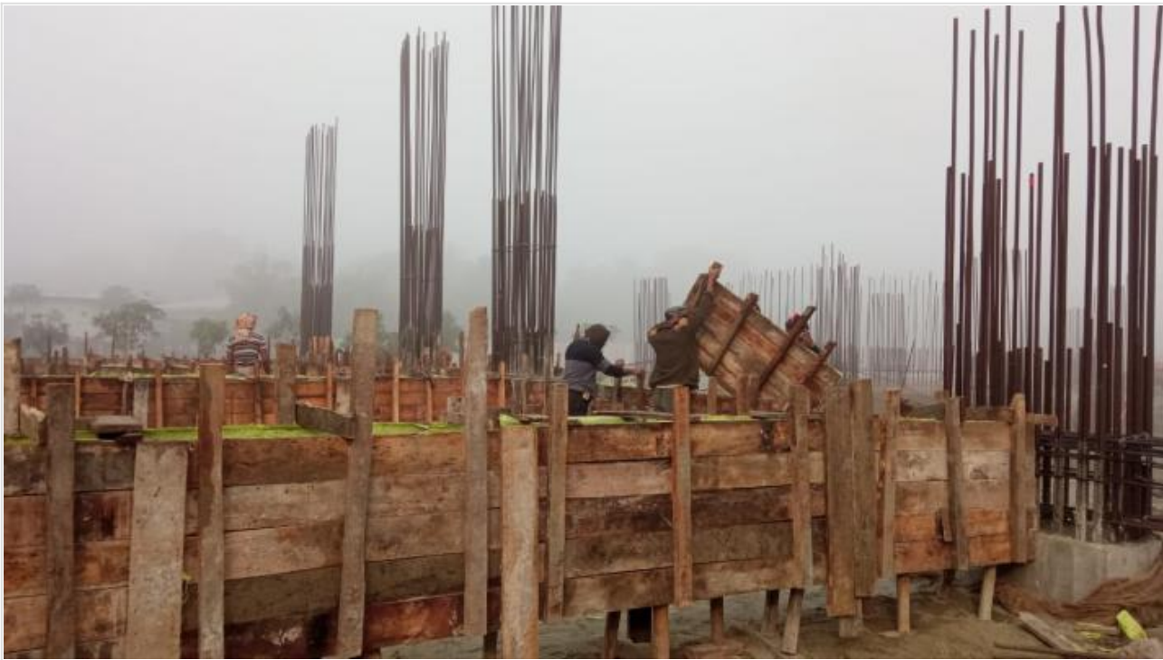
Tower-1-Grade Beam on 04-12-20
