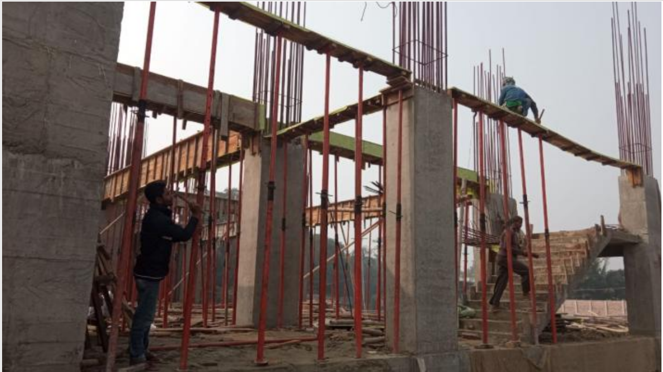
Tower-1-1st Floor Roof Beam Shuttering on 18-01-21
