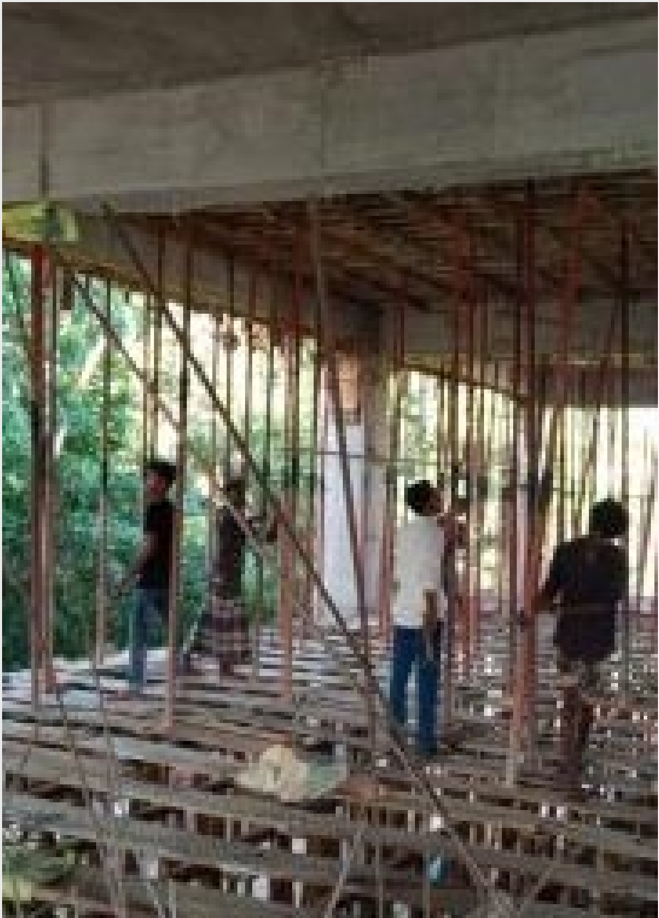
Restaurant GF Double Height Roof Slab on 24-05-21
