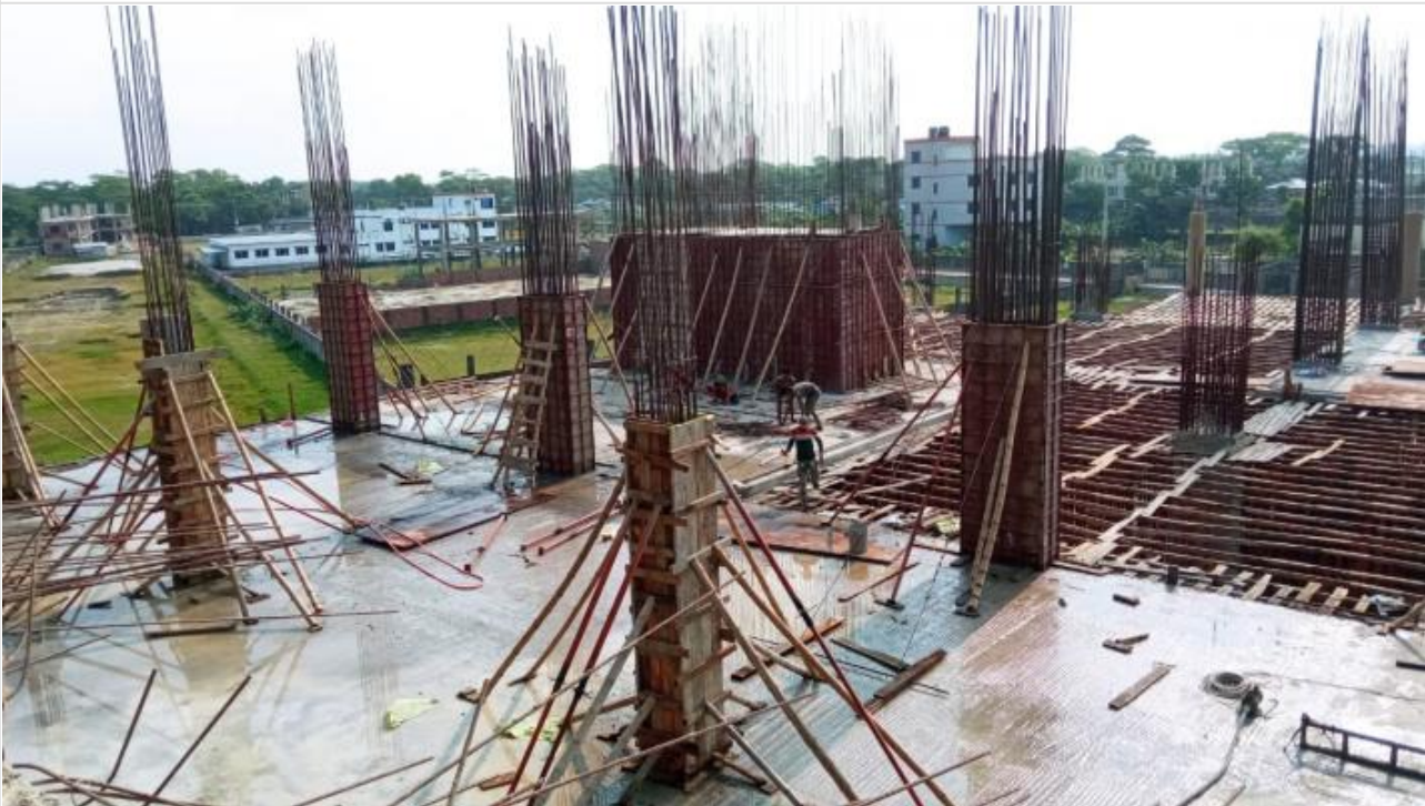
Column Concreting on 28-04-21
