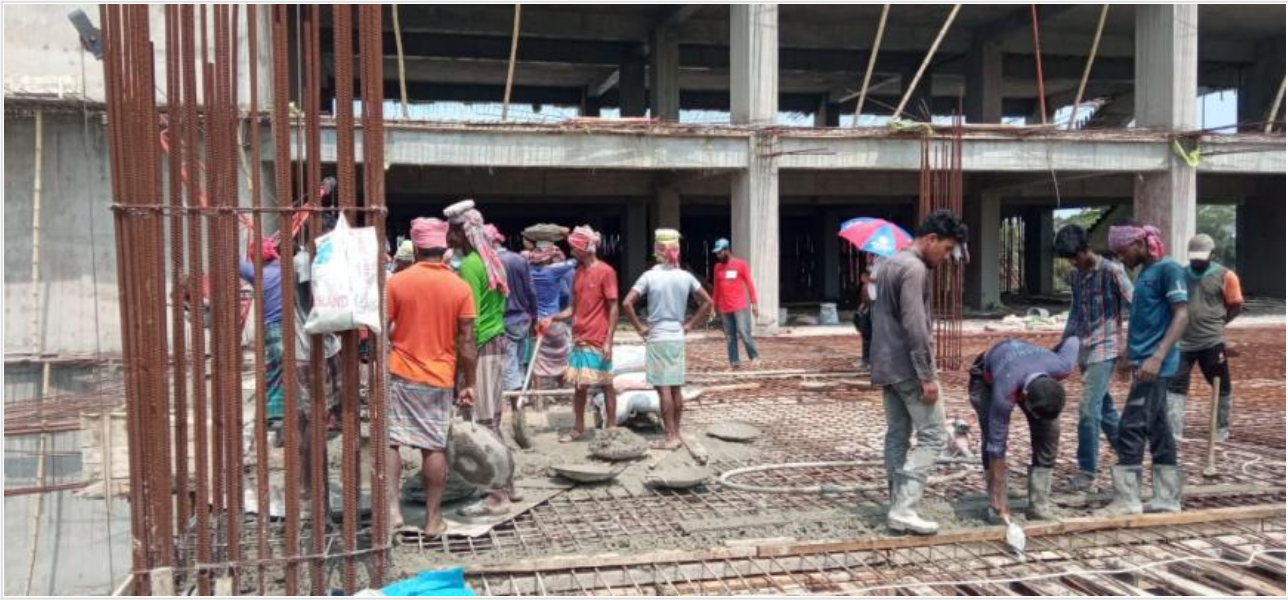
Between Tower1-2-1st Flr Roof Slab-Concr on 05-06-21
