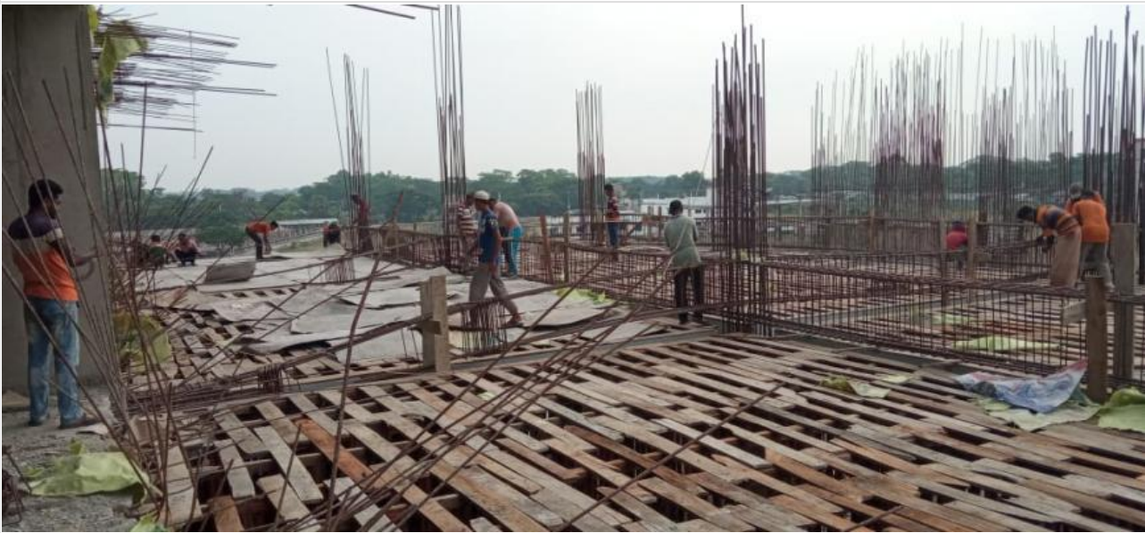
Roof Slab Shuttering on 04-05-21
