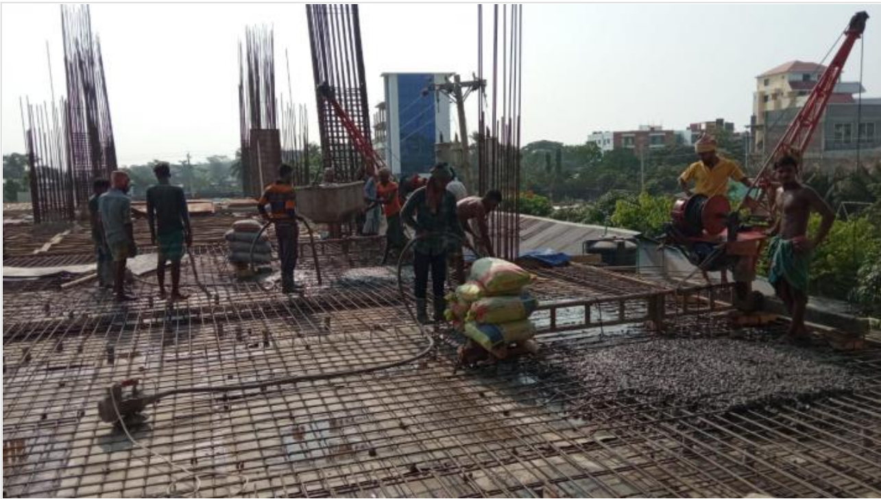
Between Tower1-2-GF Roof Slab-Concreting on 26-04-21
