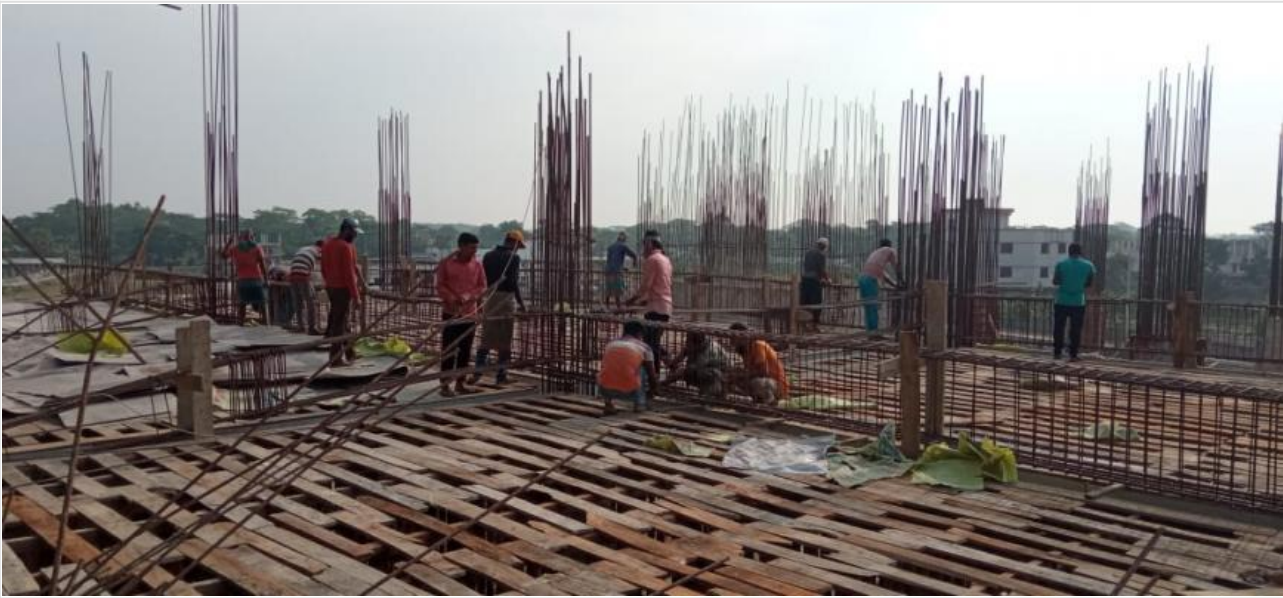
Roof Slab Shuttering on 04-05-21
