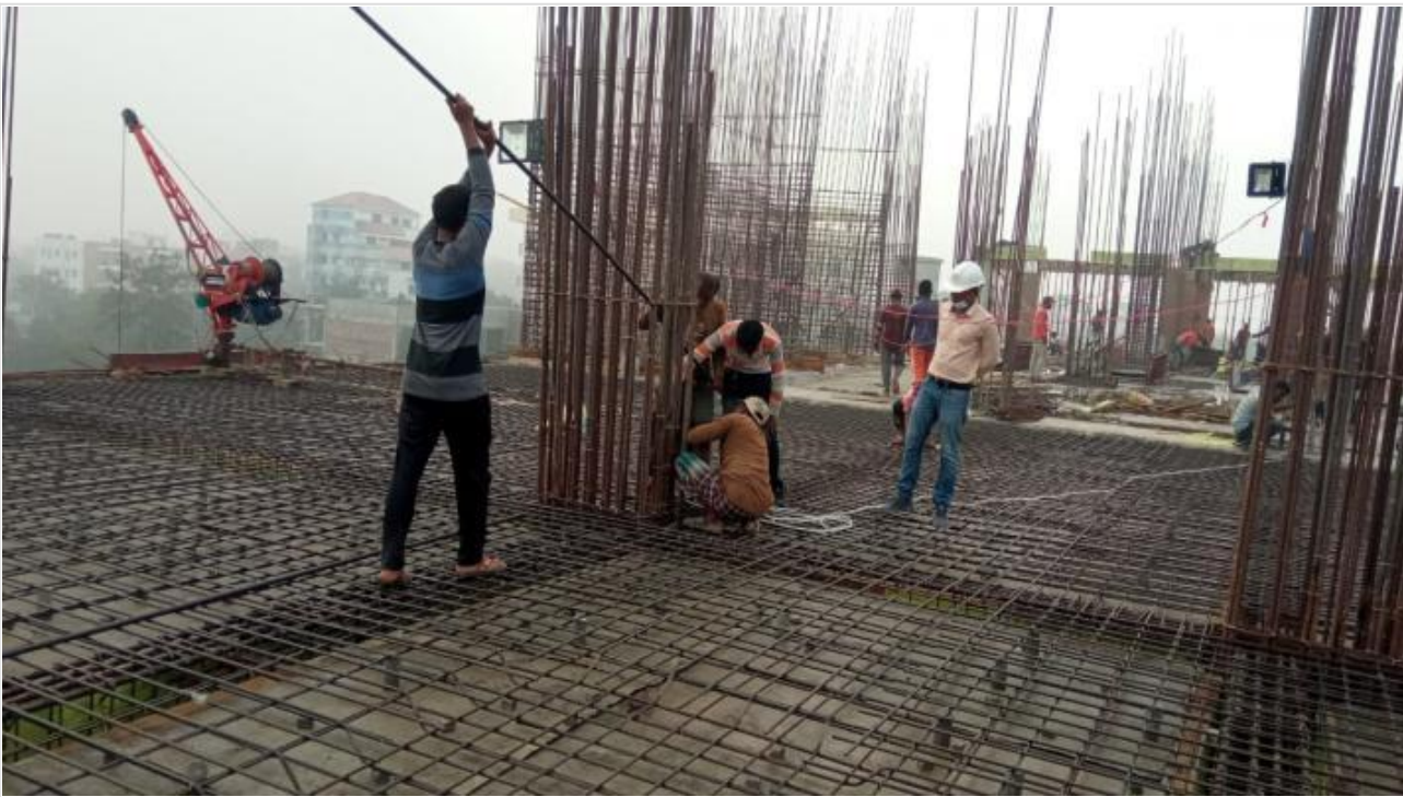
Tower-1-2nd Floor Roof Inspection on 25-02-21
