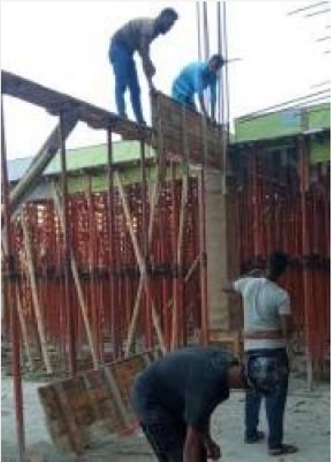
Roof Beam Shuttering on 09-05-21
