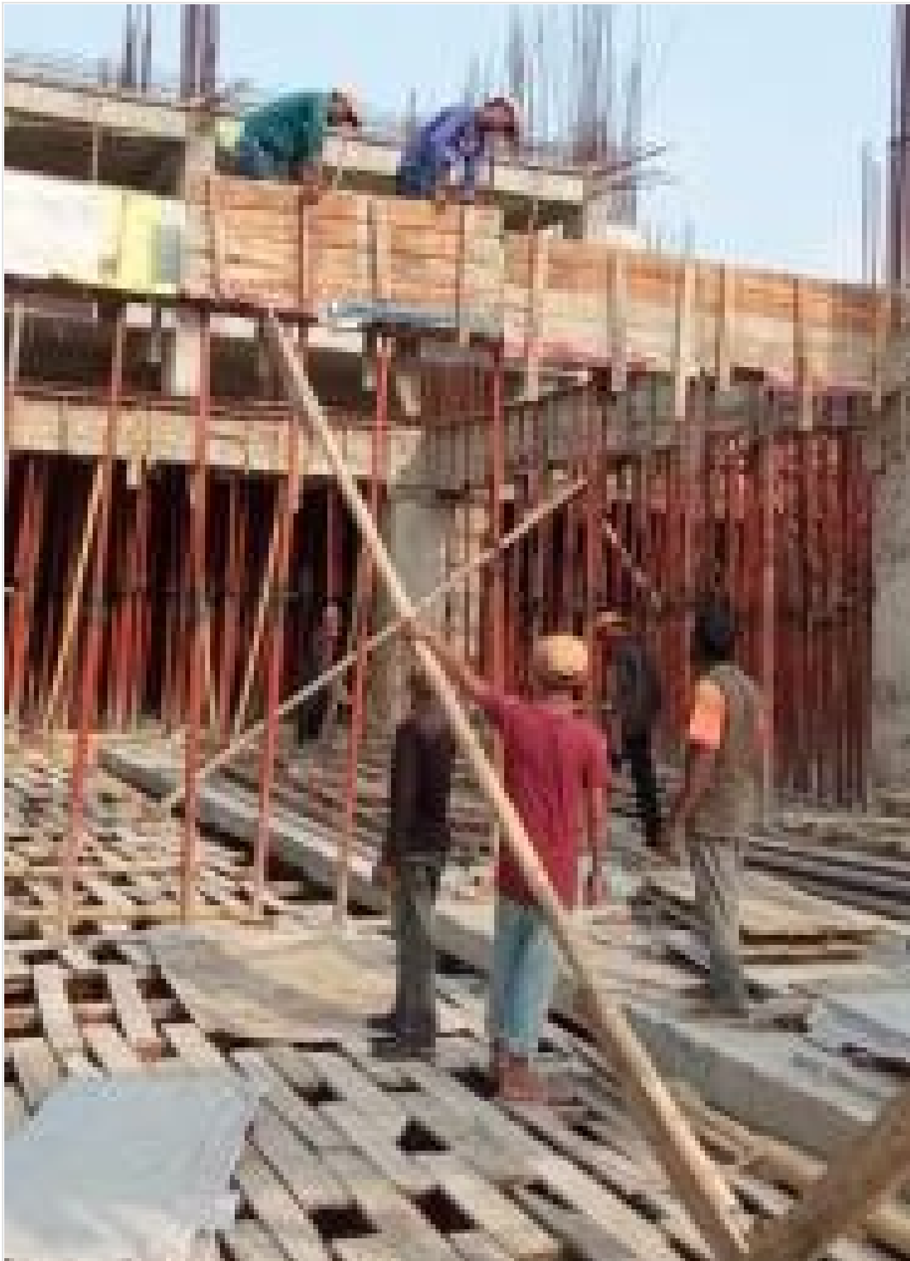
Beam Shuttering on 31-05-21
