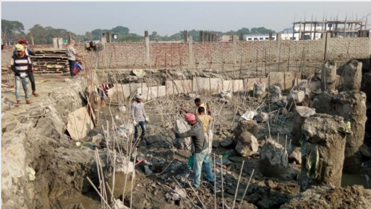
Tower-2-Pile Head Breaking on 27-12-20
