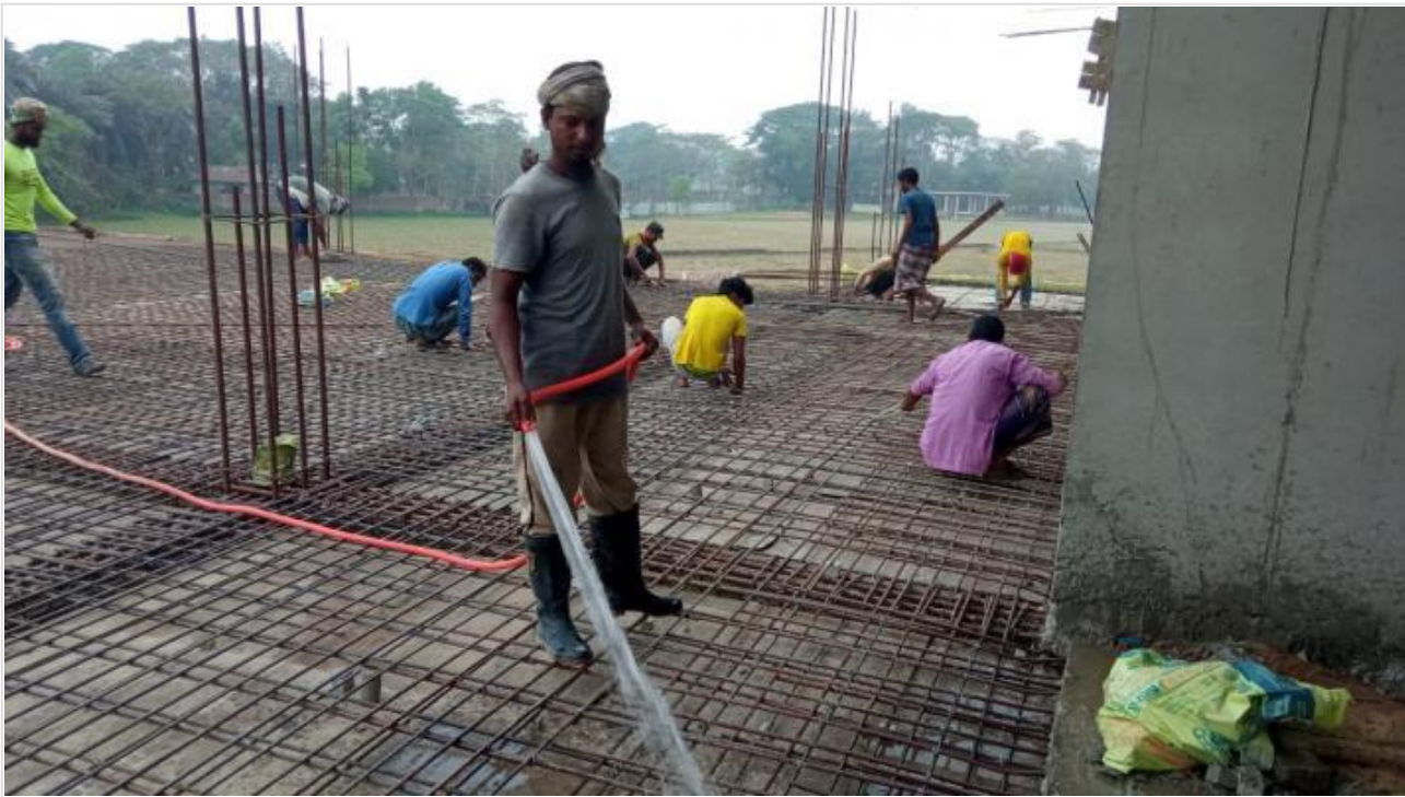
Restaurant-Double Height Slab Concreting on 02-03-21
