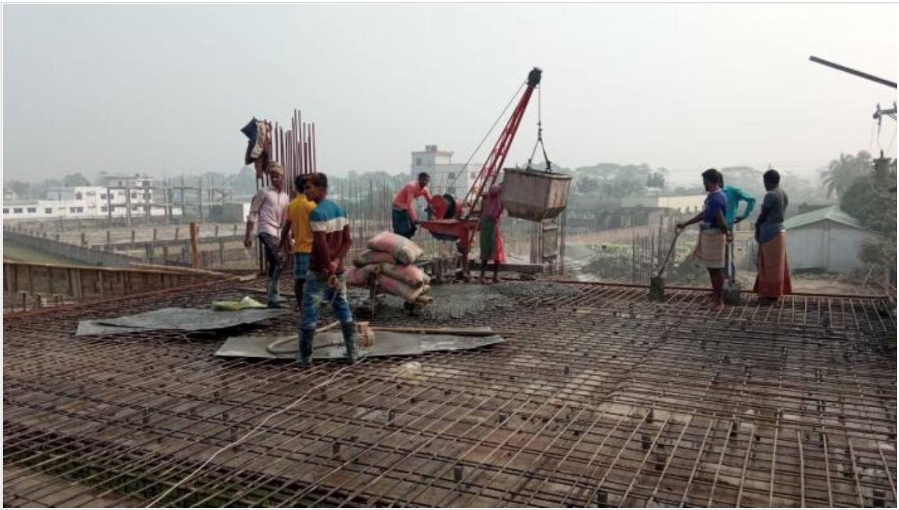
Tower-1-GF Roof Slab 1800 sft Concreting on 18-01-21
