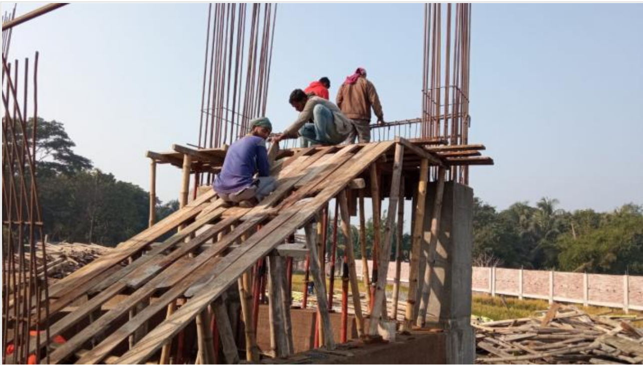
Tower-1-GF Stair Shuttering on 27-12-20
