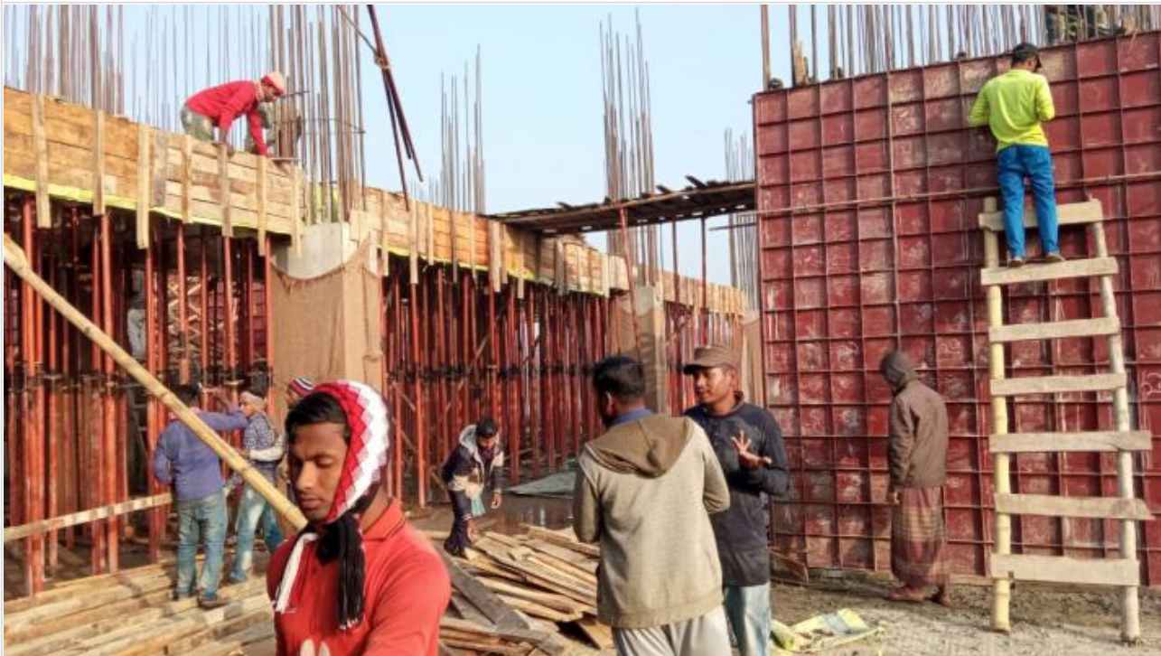
Tower-1-Lift Core and Slab Shuttering on 27-01-21
