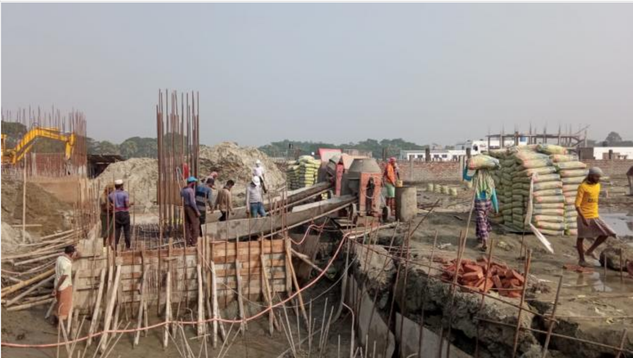
Tower-1-Pilecap Concreting on 12-12-20
