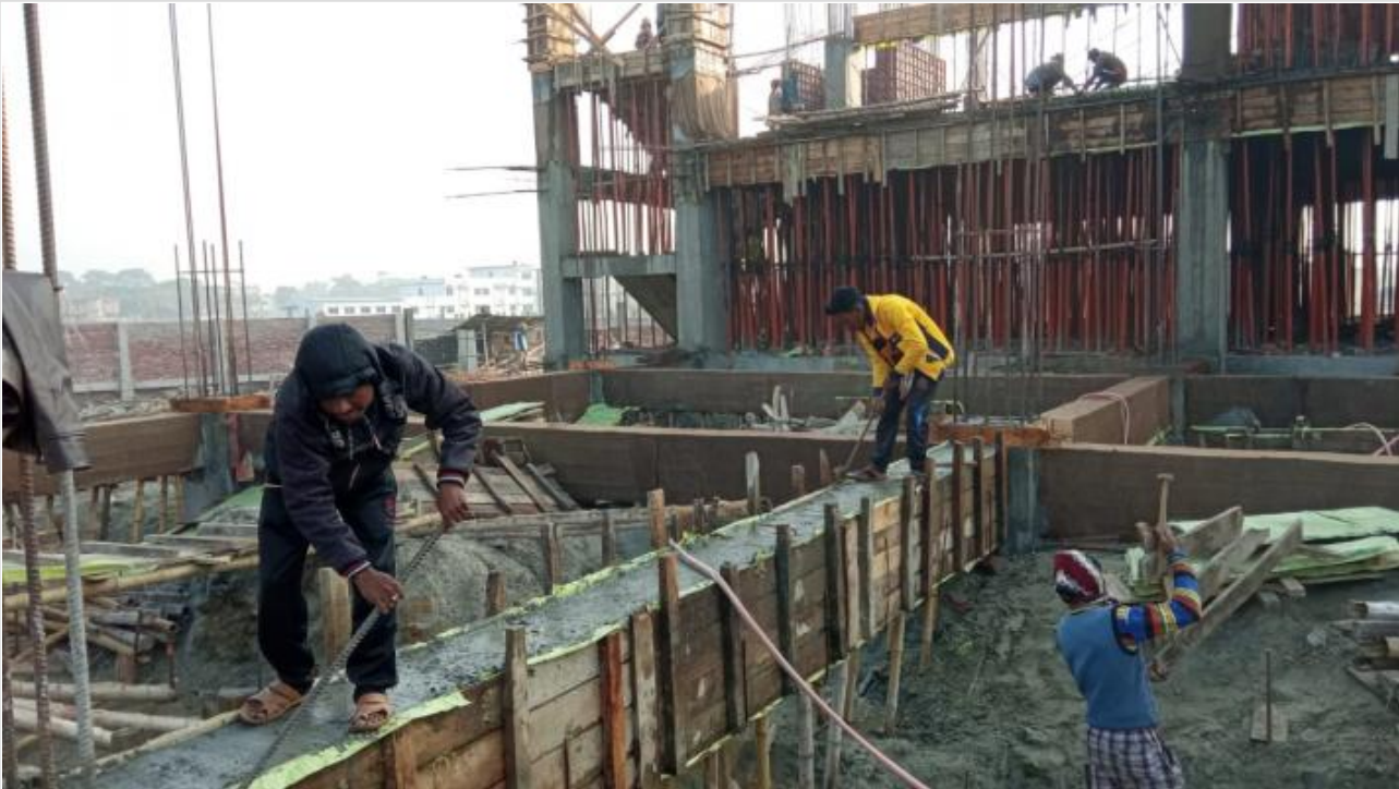
Tower-2-GB Shutter Removing on 05-02-21
