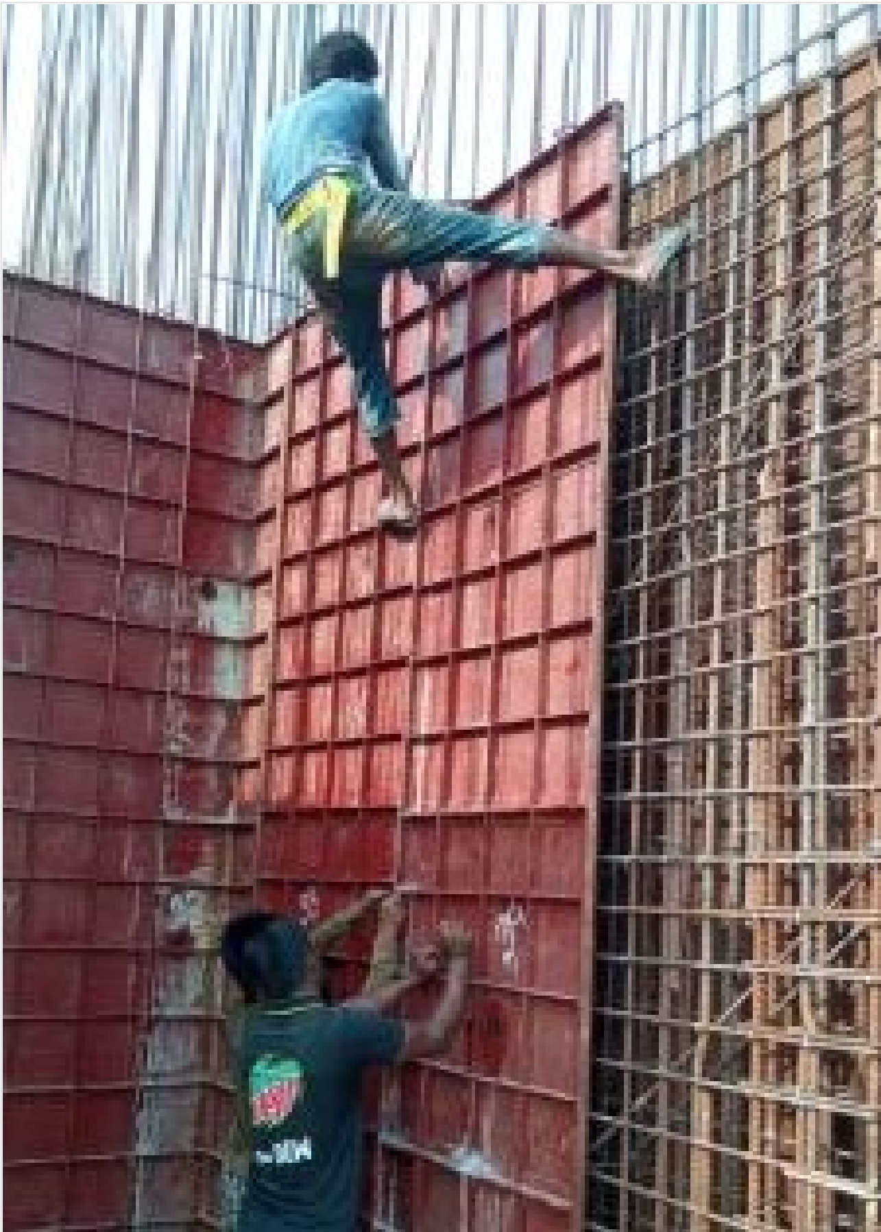
Lift Core Wall Shuttering on 26-04-21
