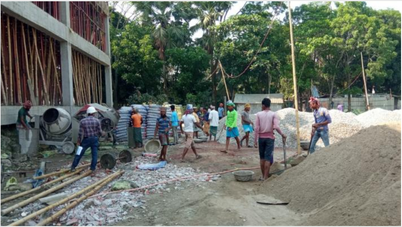
Restaurant GF Doubl Ht Slab-1-4/A-B-Conc on 24-04-21
