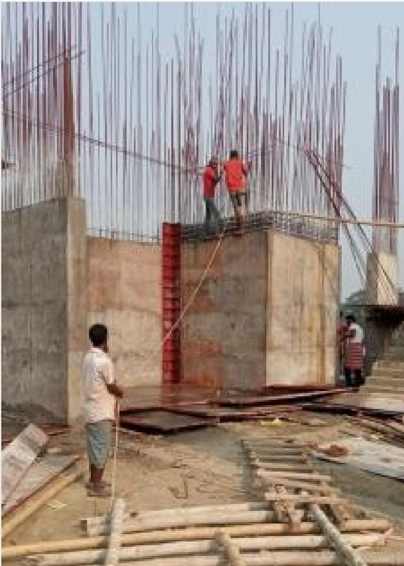
Tower-2: Lift Wall De-shuttering Work on 25-03-21
