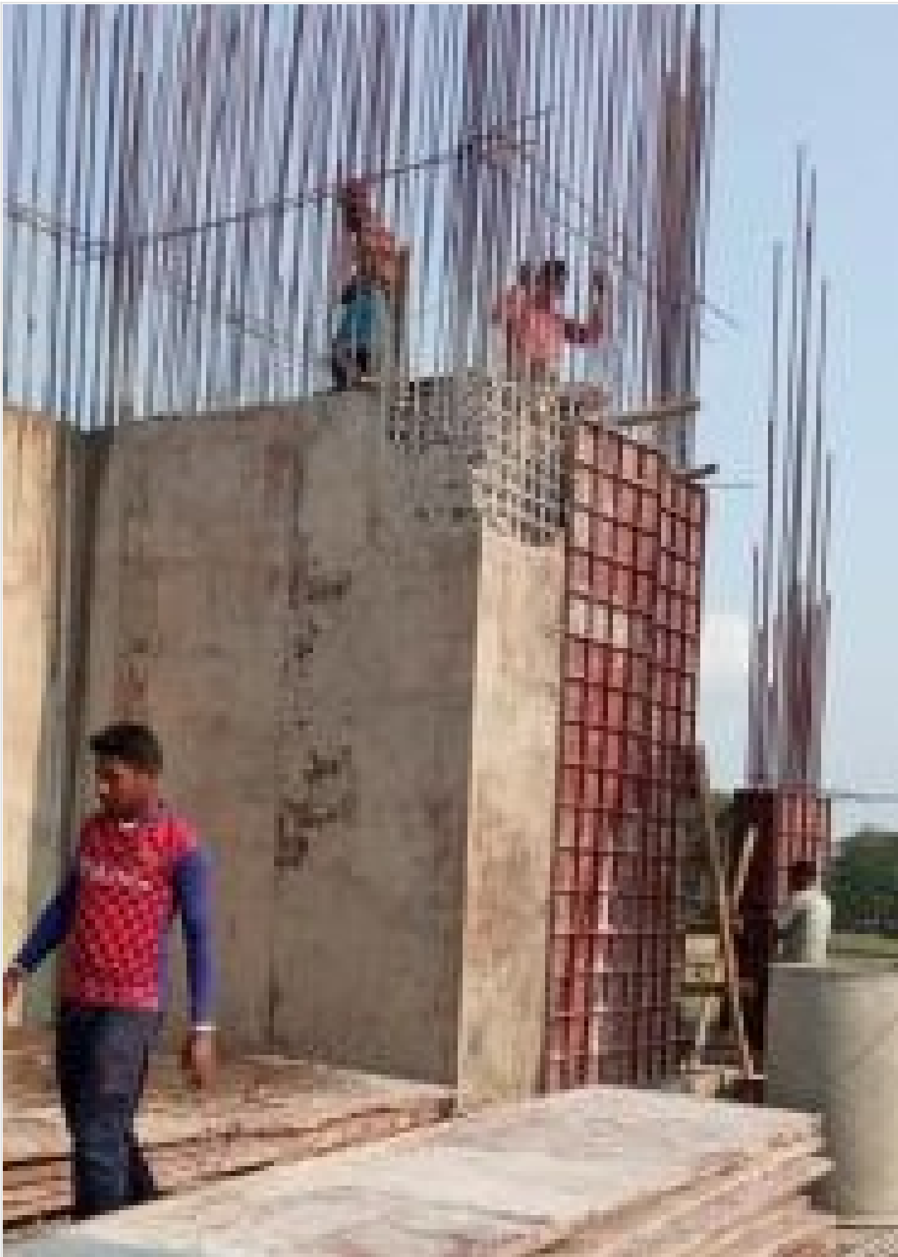
Tower-2-Lift Core Deshuttering on 02-05-21
