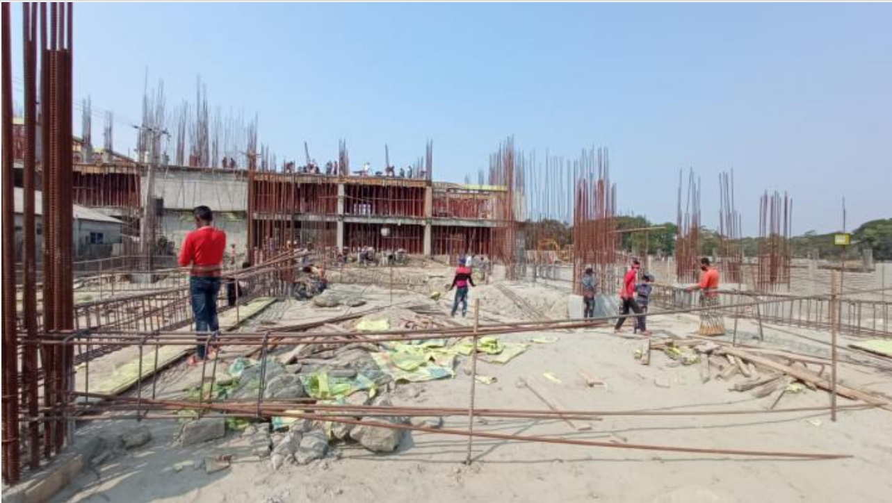
Tower-1-1st Floor Roof Slab Concreting on 07-02-21
