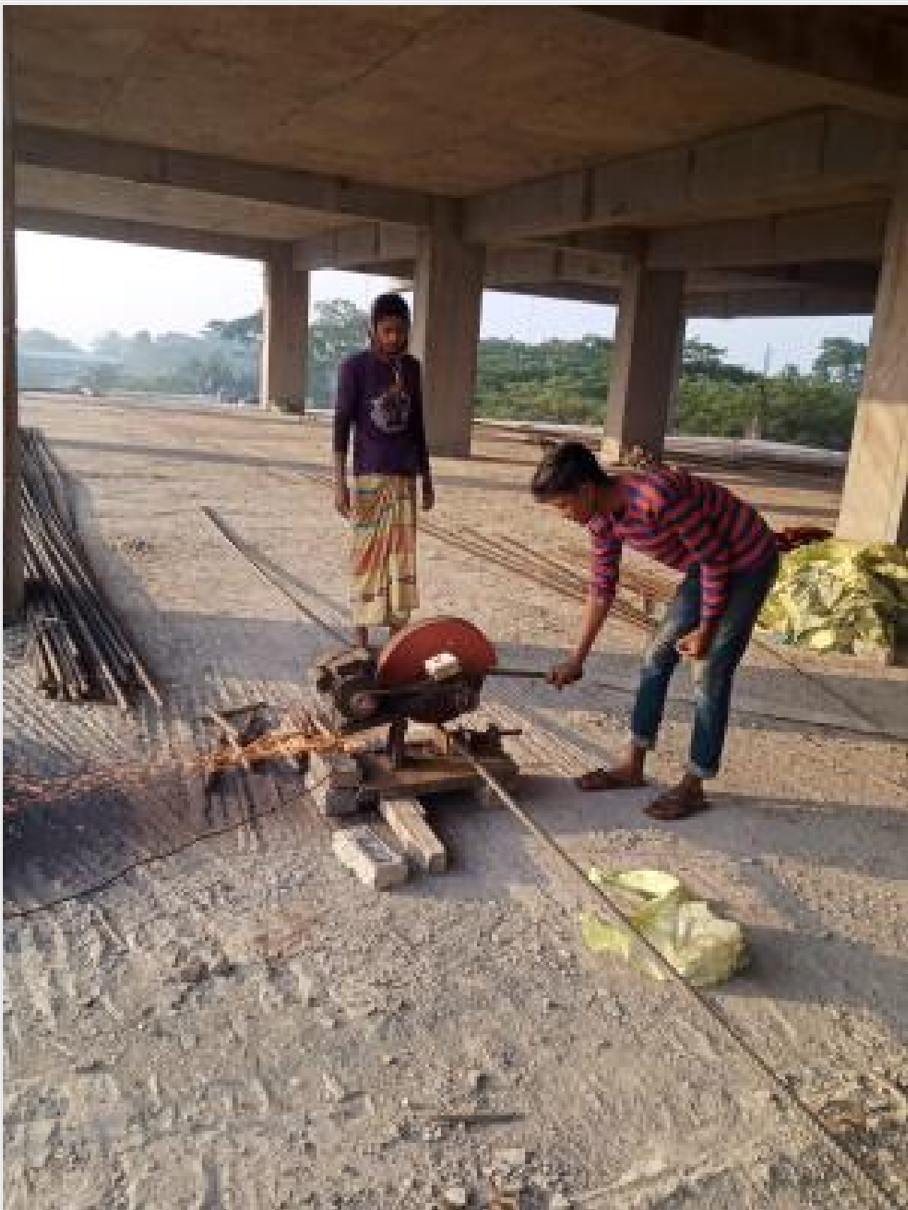
Re-bar Cutting on 08-01-22
