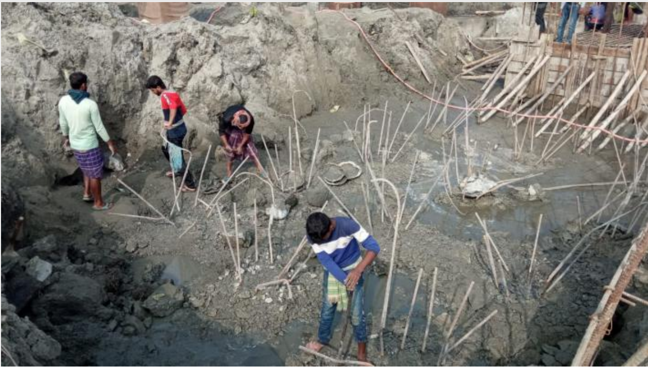
Tower-1-Pile Cap Re-bar Fabrication on 12-12-20
