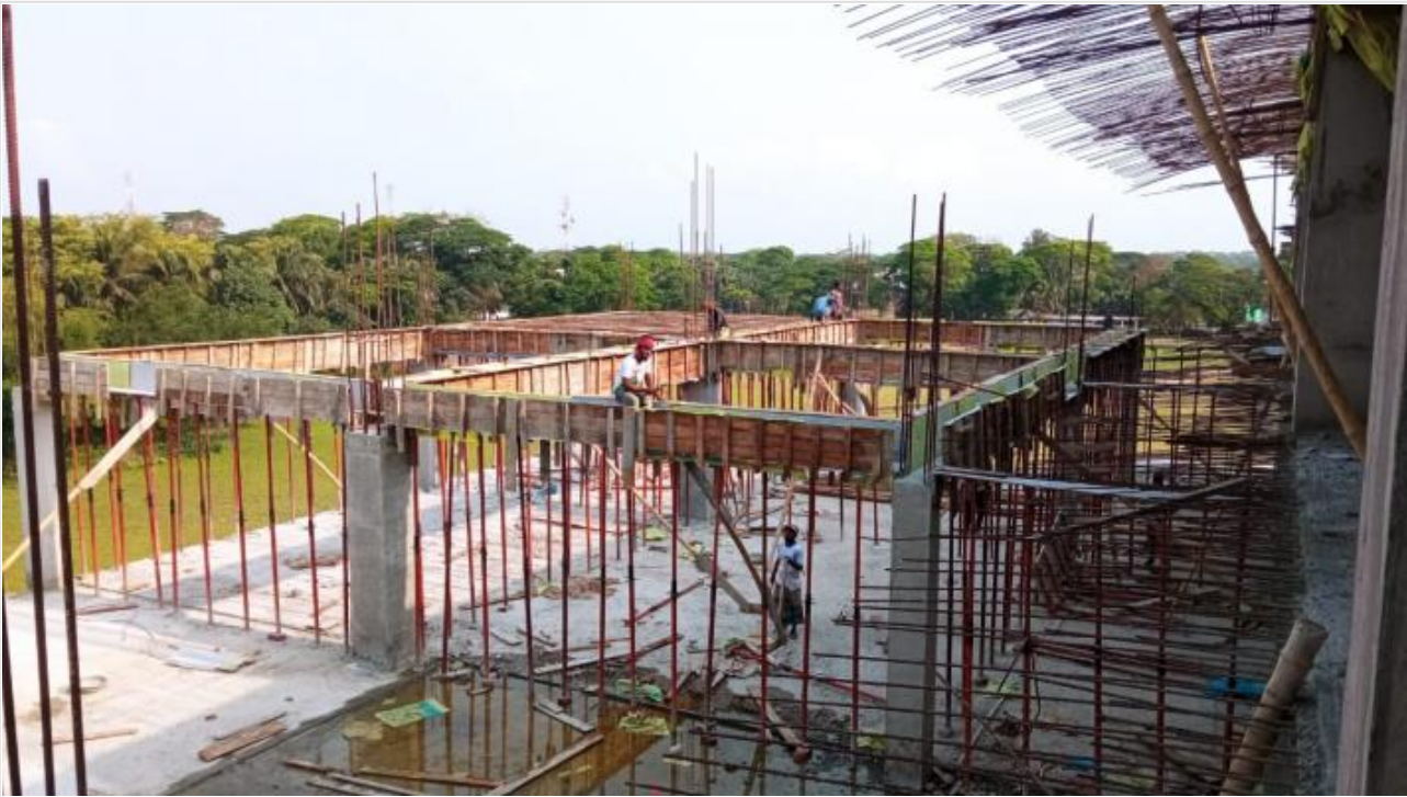
Beam Shuttering on 28-04-21
