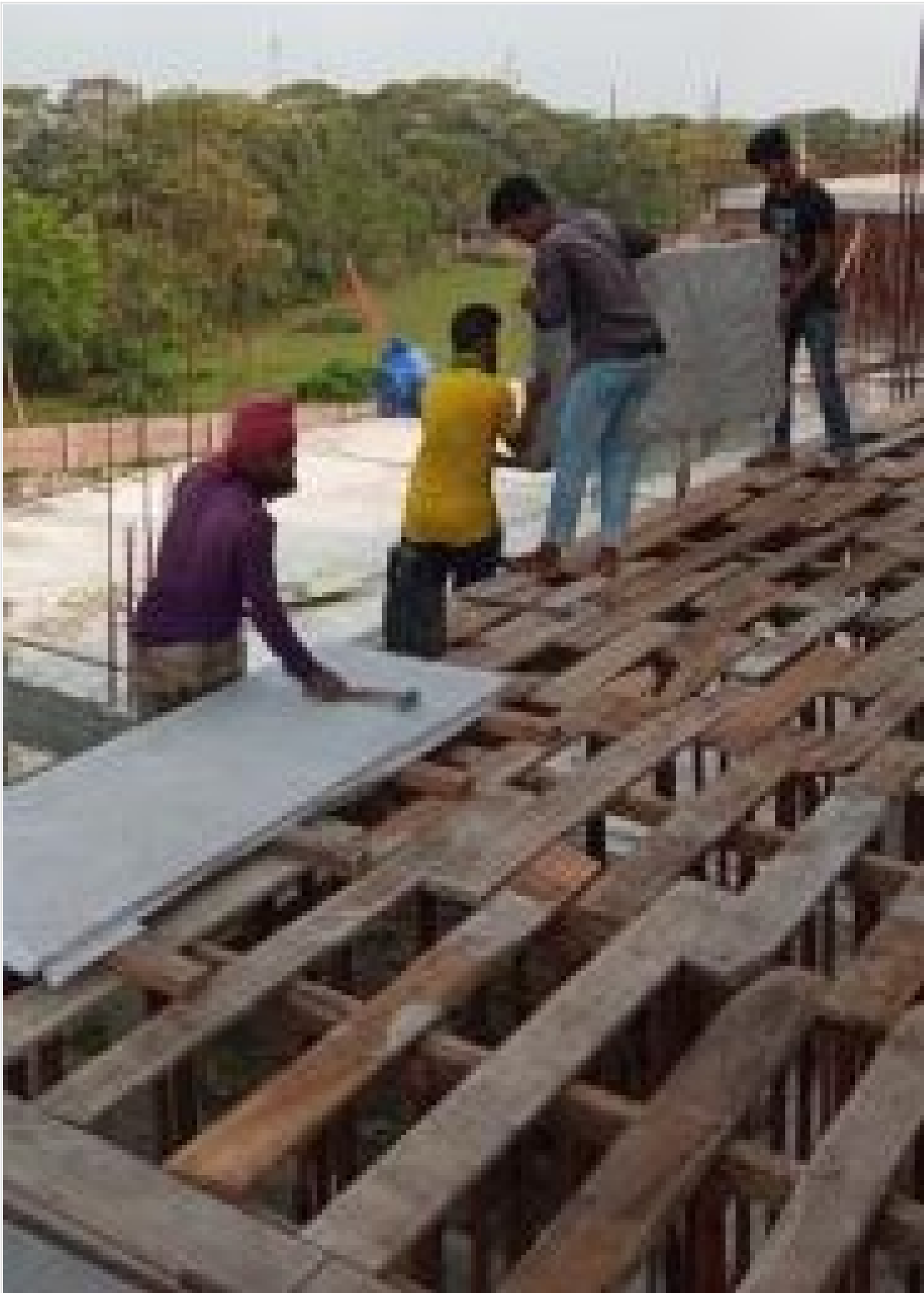
Slab Shuttering on 31-05-21
