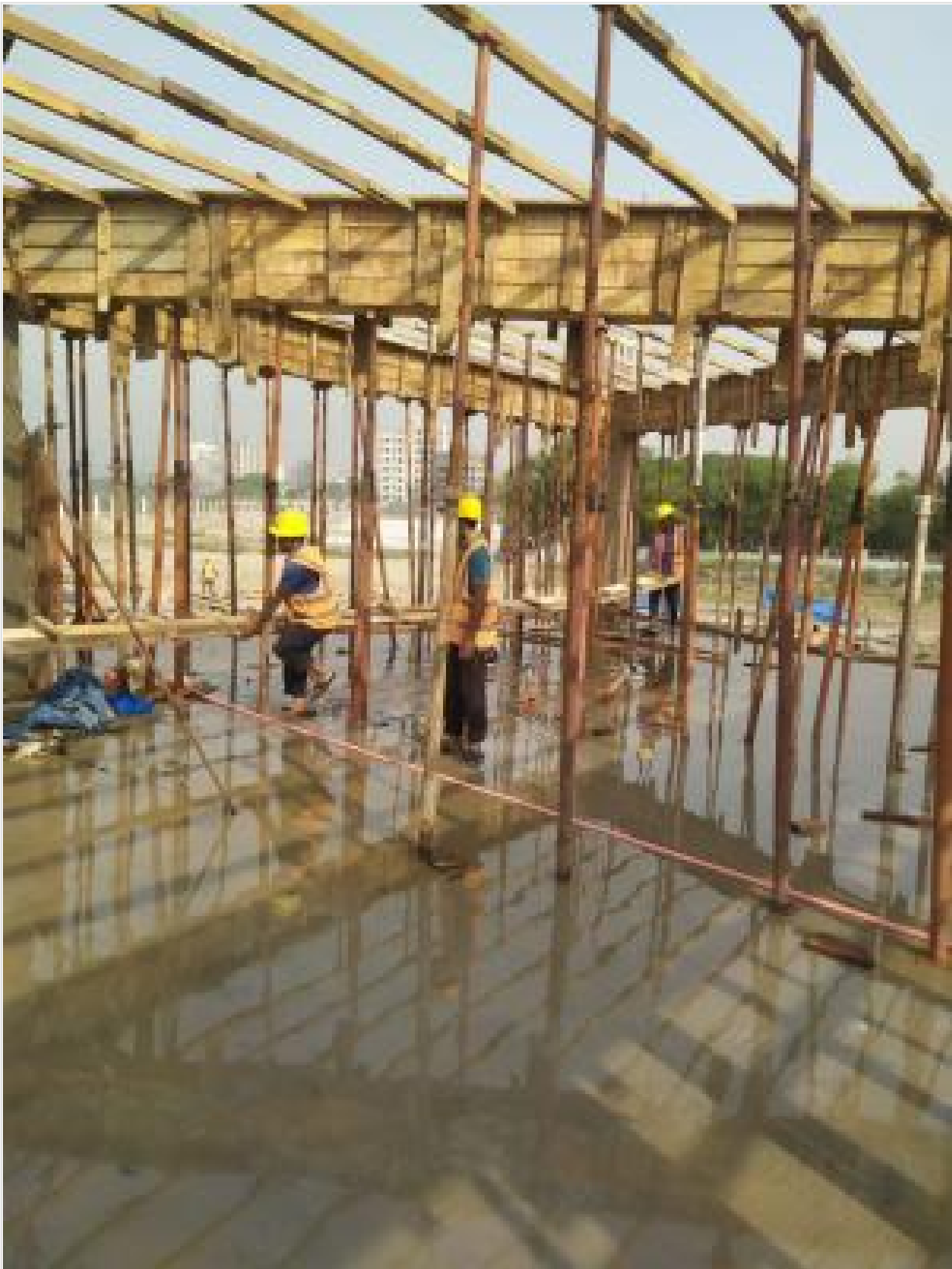
Mosque 1st Floor Slab Shuttering on 27-03-21
