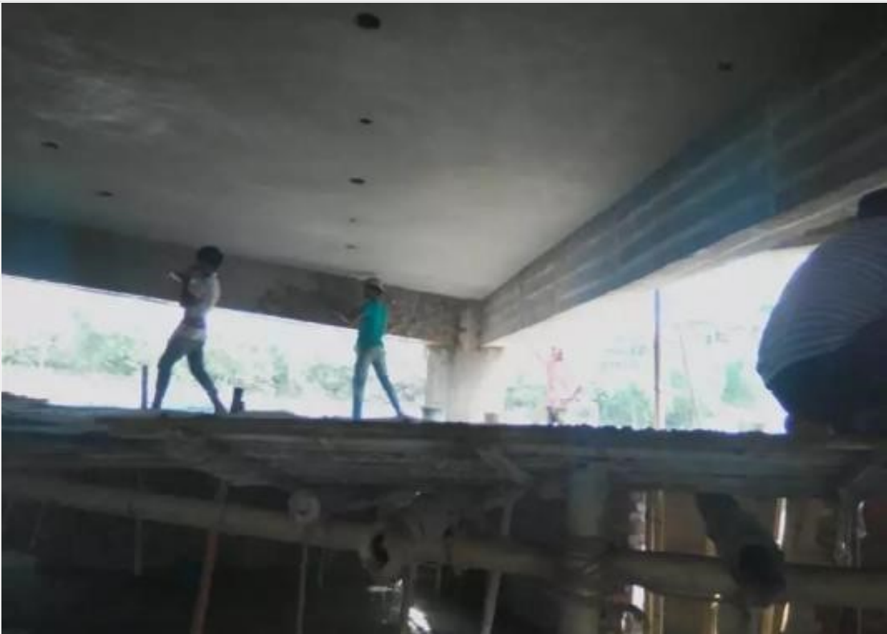
Mosque-Basment Plaster Work on 14-04-21
