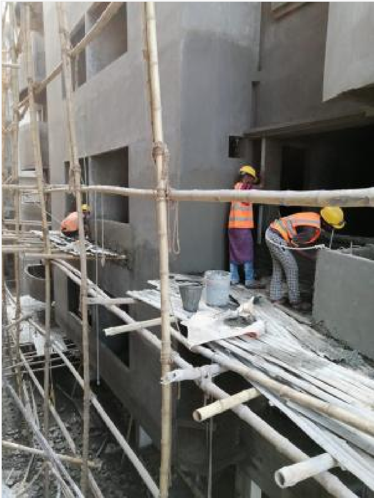
Bulding-Q-Out-side Plastering on 09-05-21
