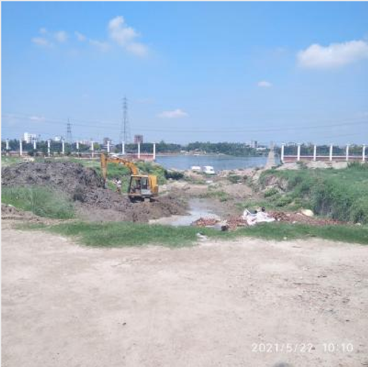
Landing Station-Excavation on 22-05-21
