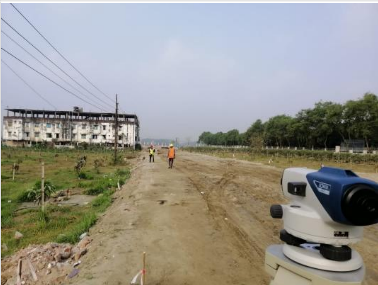
40 ft Road Dressing and Levelling on 01-03-21
