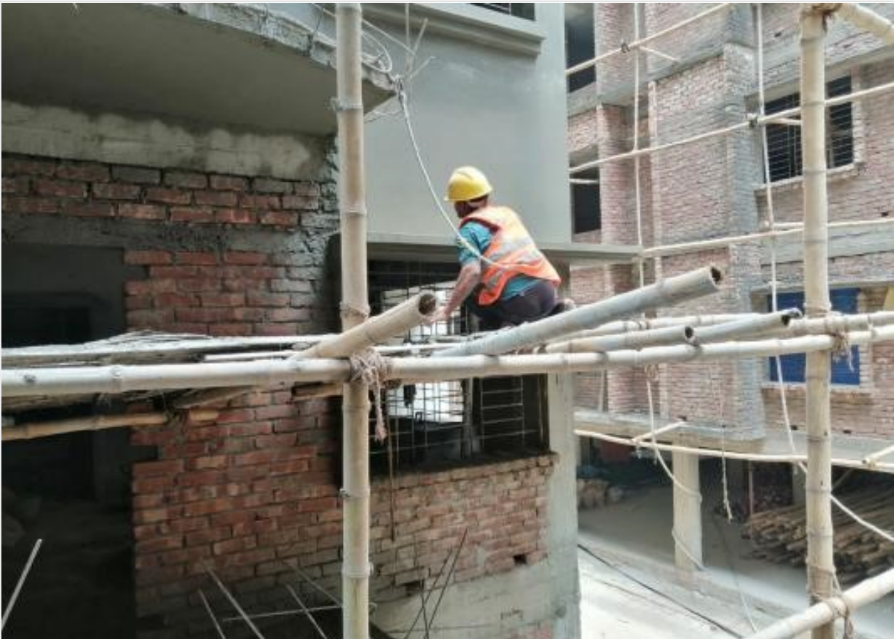
Out-side Plastering on 22-04-21
