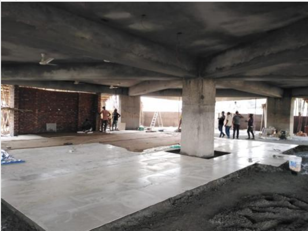
Mosque-Basement Tiles Work on 11-04-21
