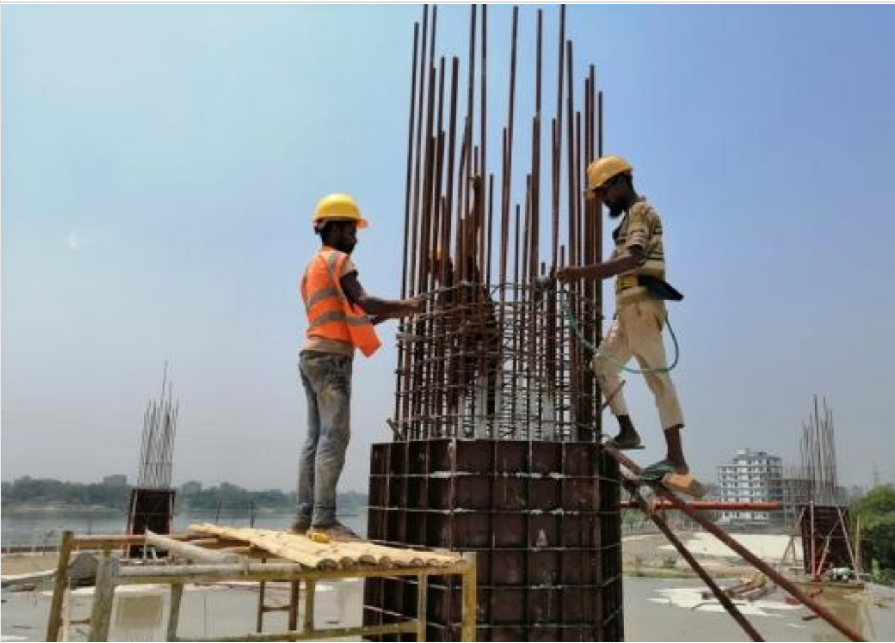
Mosque-1st Floor Column Re-bar Work on 19-04-21
