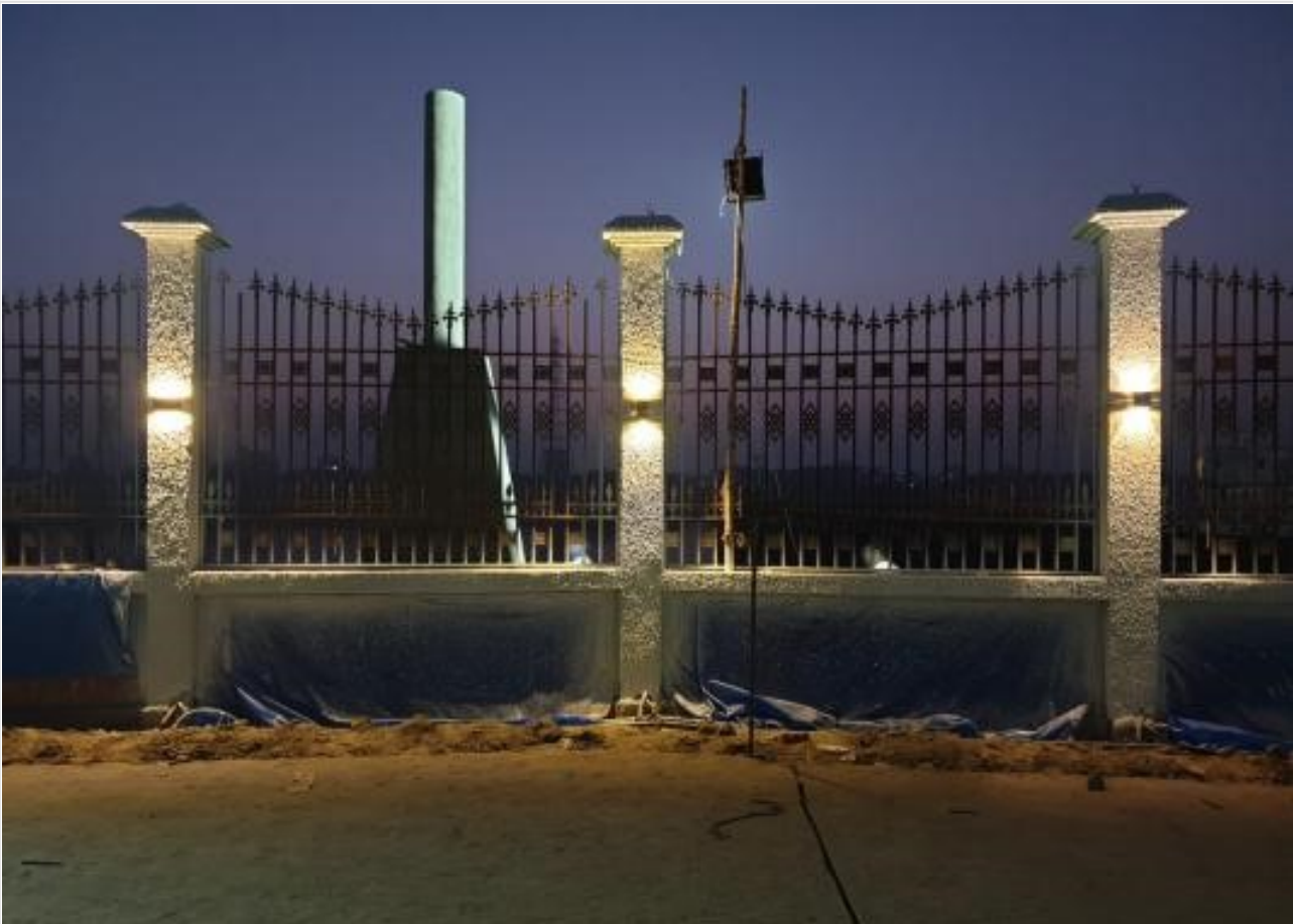
Riverside Bontile Rectification & Lighti on 01-02-21
