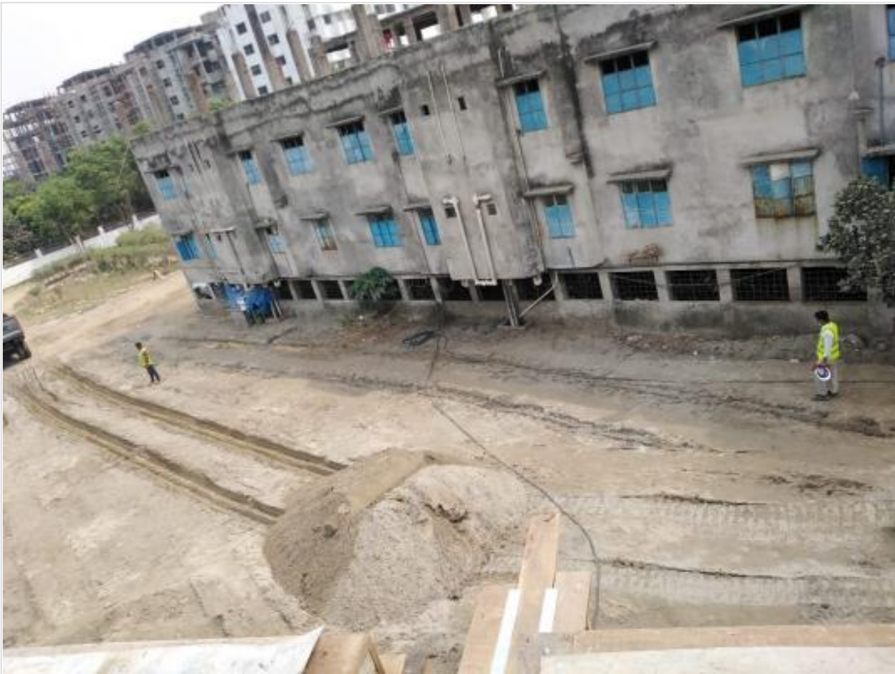
Mosque-20ft Connecting Road-Filling on 31-03-21
