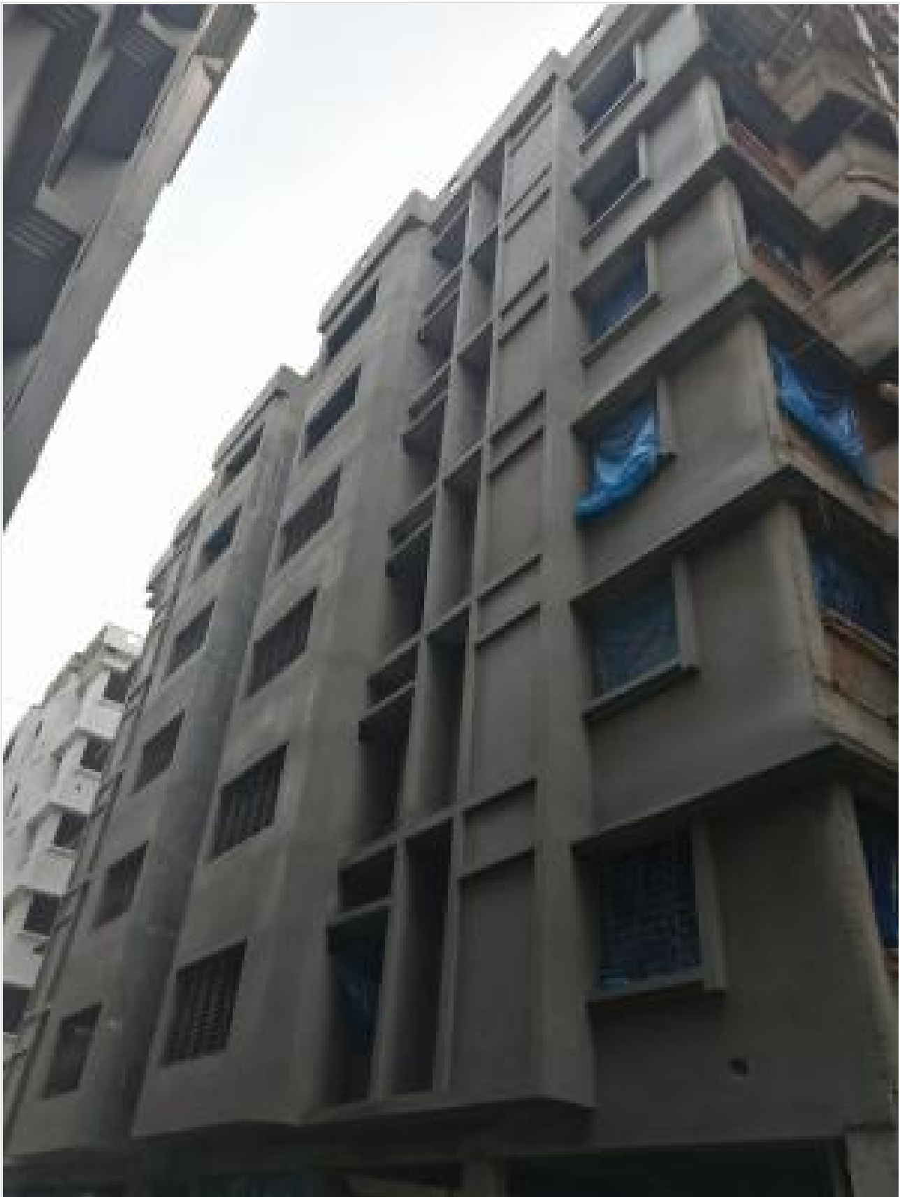
Building-J outside plastering on 28-01-21
