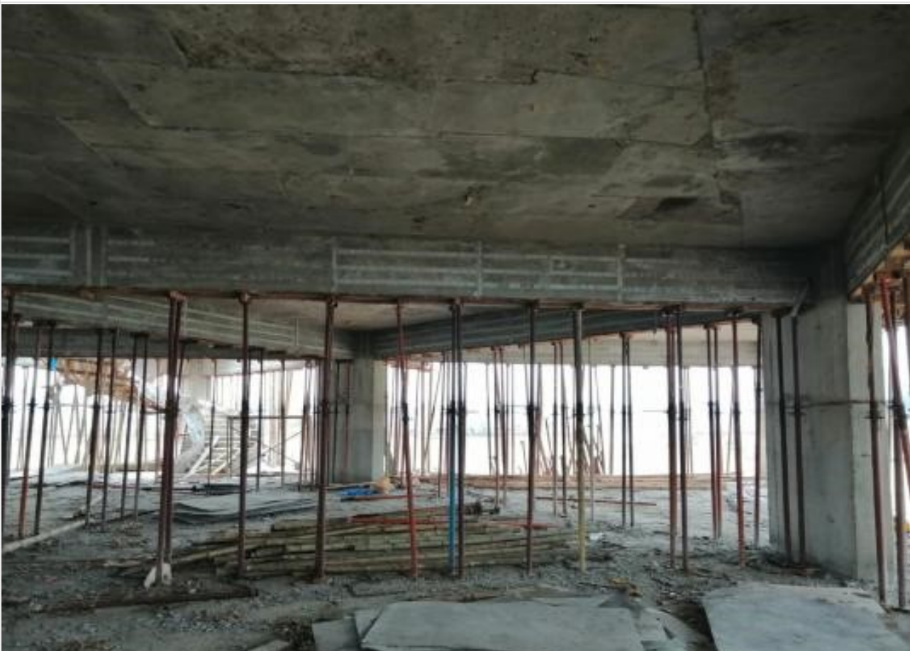
Mosque-Ground Floor-Roof Slab de-shutter on 22-04-21
