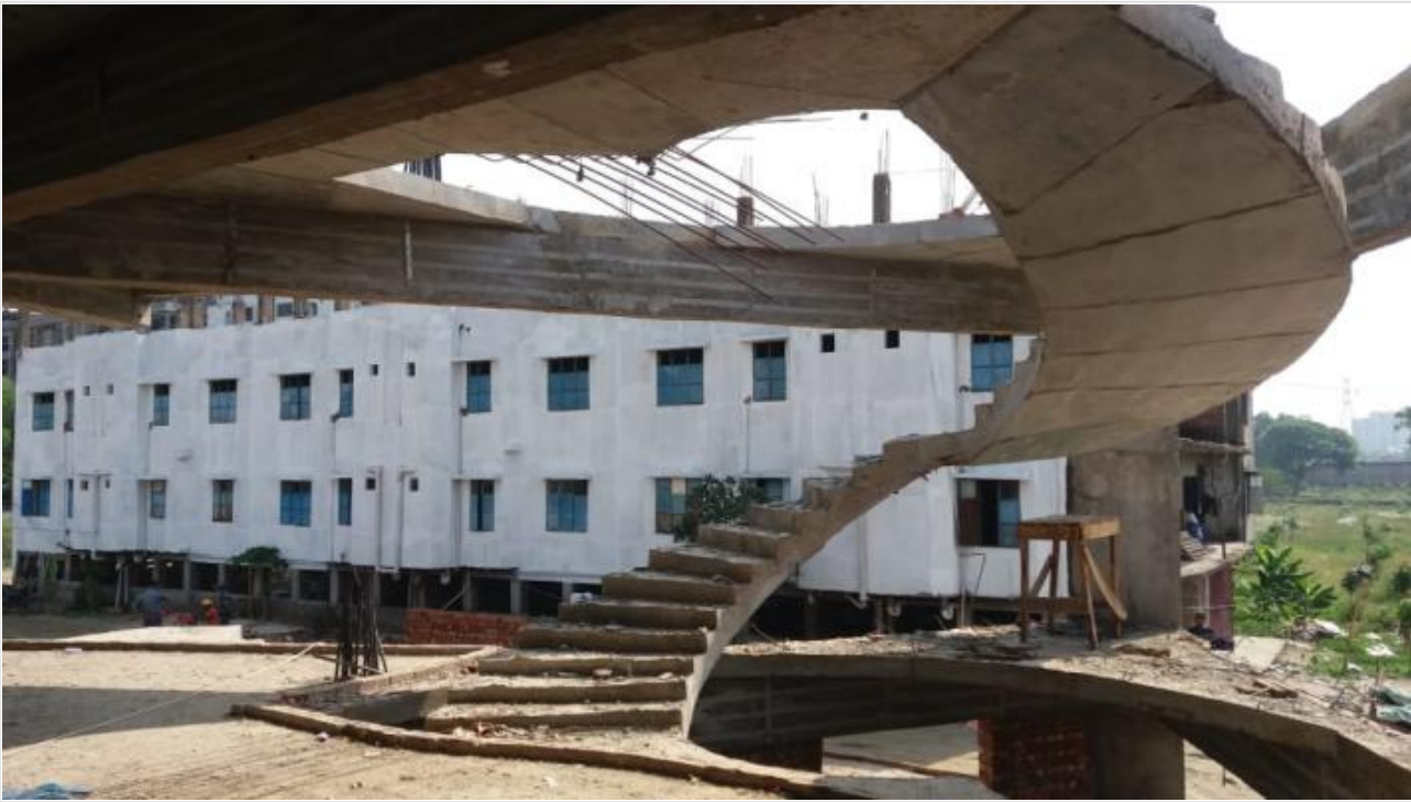
Mosque-Stair Case on 25-04-21
