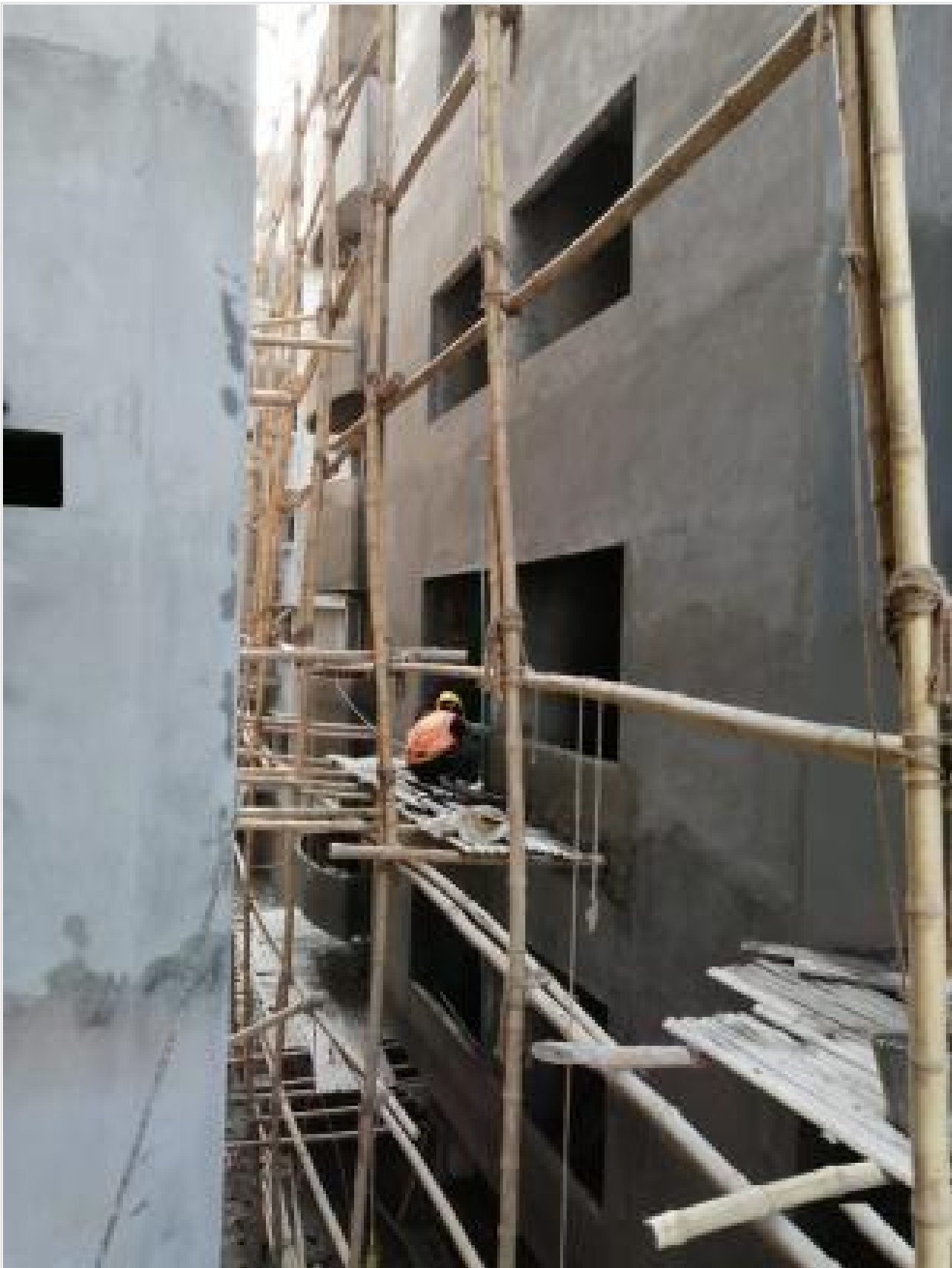
Bulding-Q-Out-side Plastering on 09-05-21
