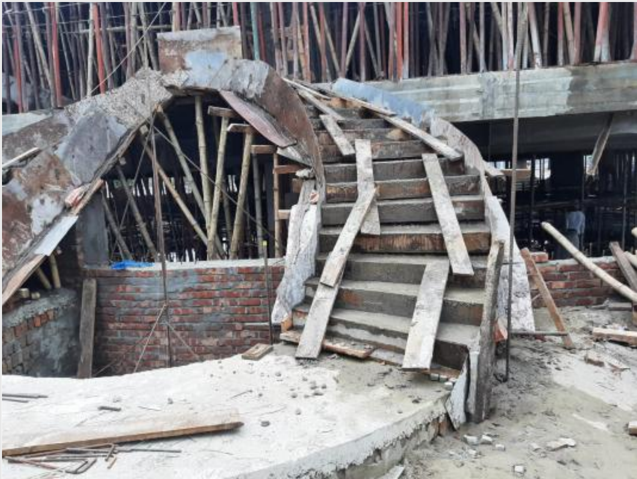
Mosque-Esatside Stair Case on 11-04-21
