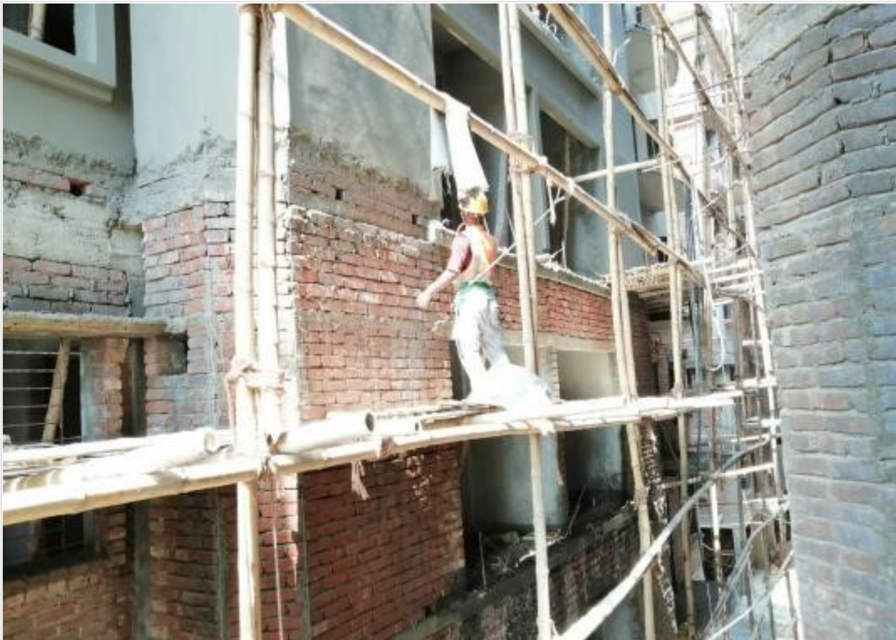
Out-side Plaster Work on 20-04-21
