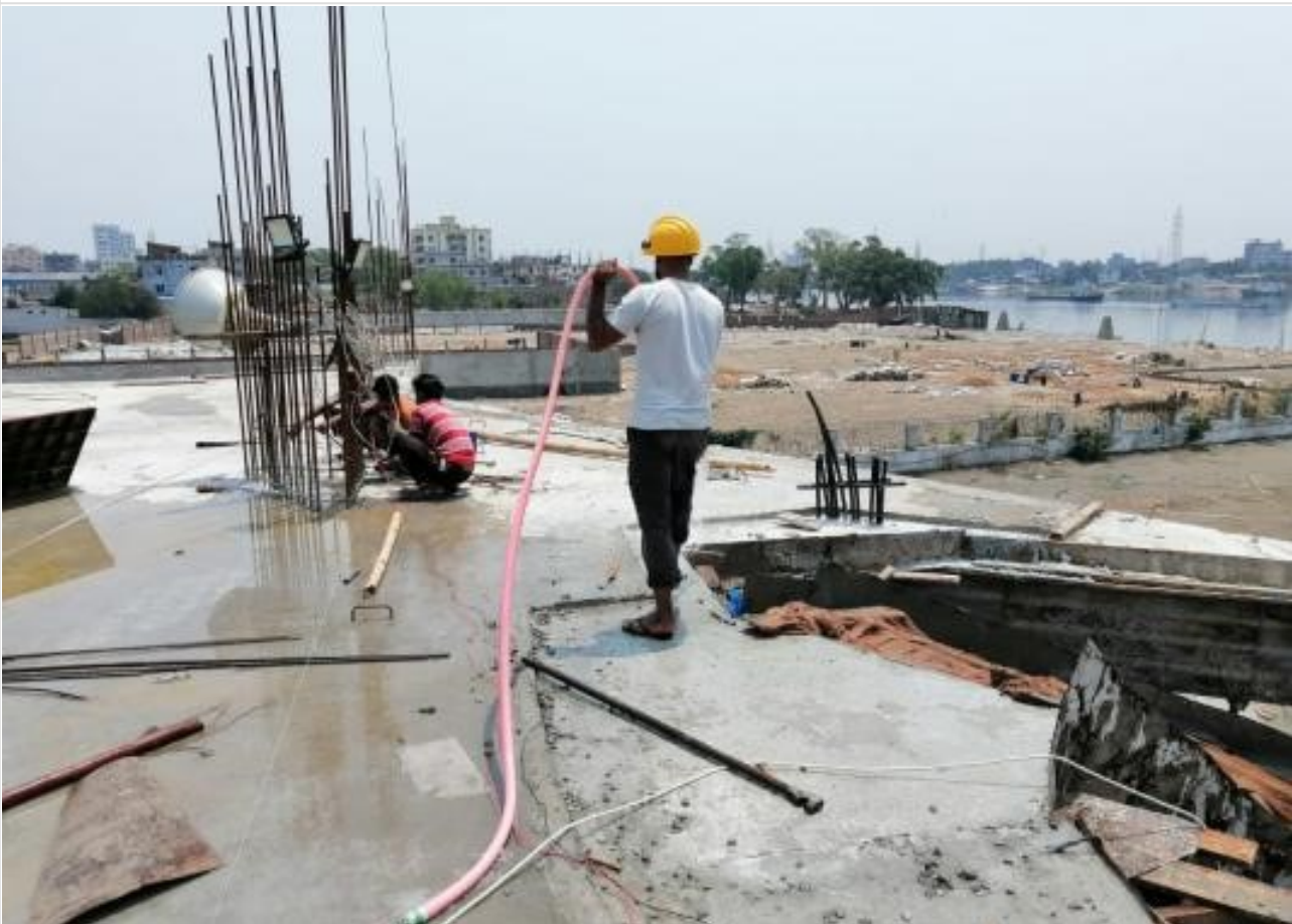
Mosque-Basement-Ancillary Work on 16-04-21
