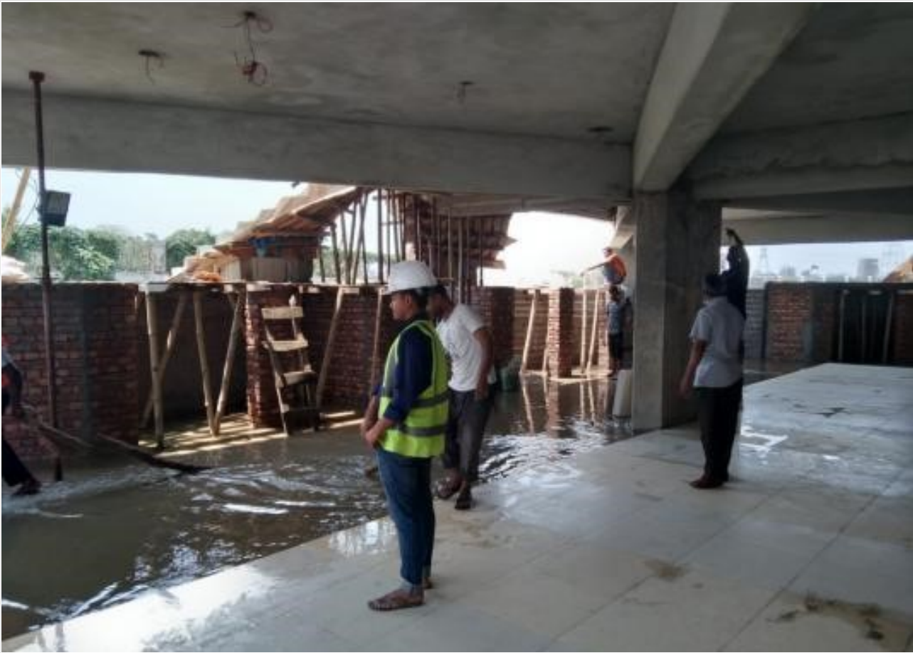
Mosque-Basement-Ancliary Work on 17-04-21
