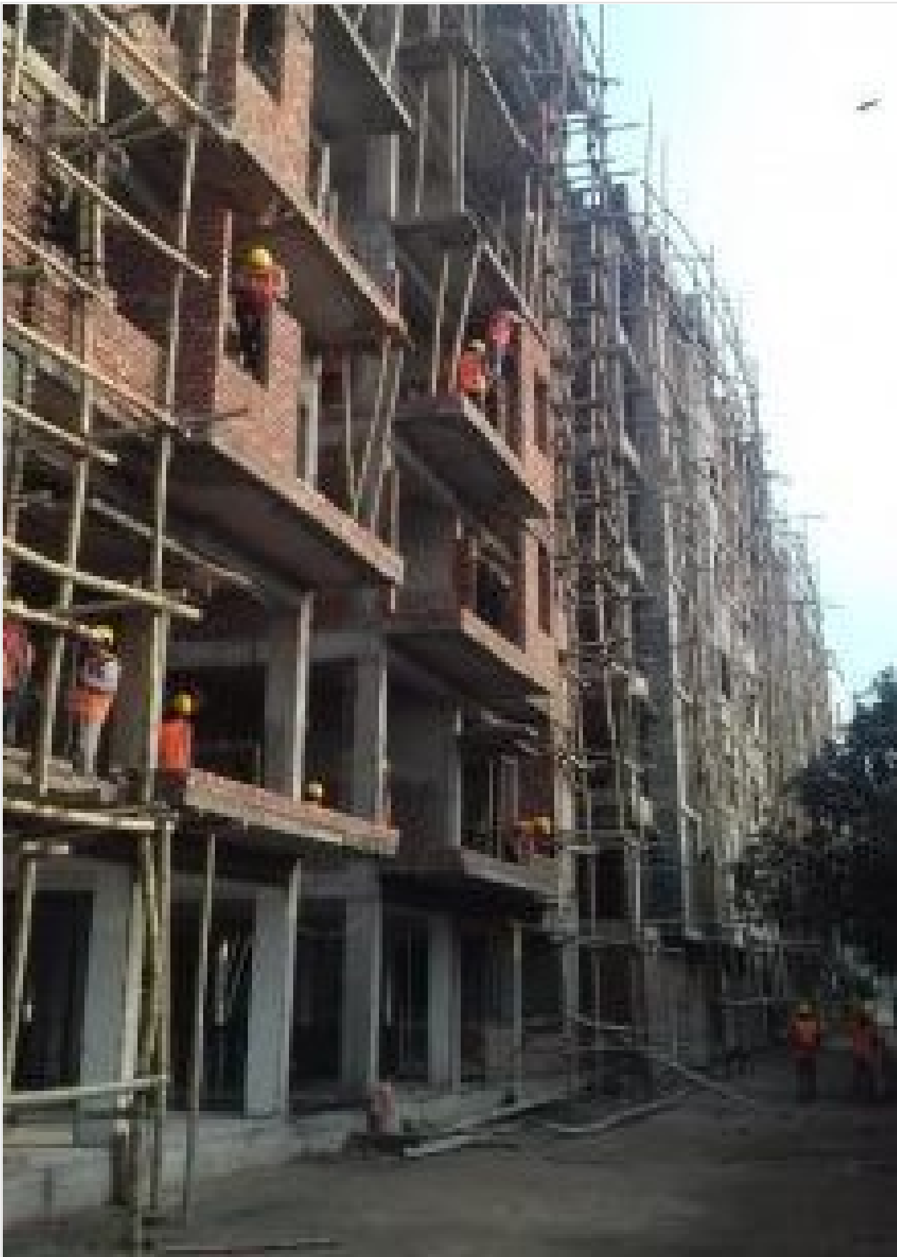
Scaffolding for outside plastering Build on 29-01-21
