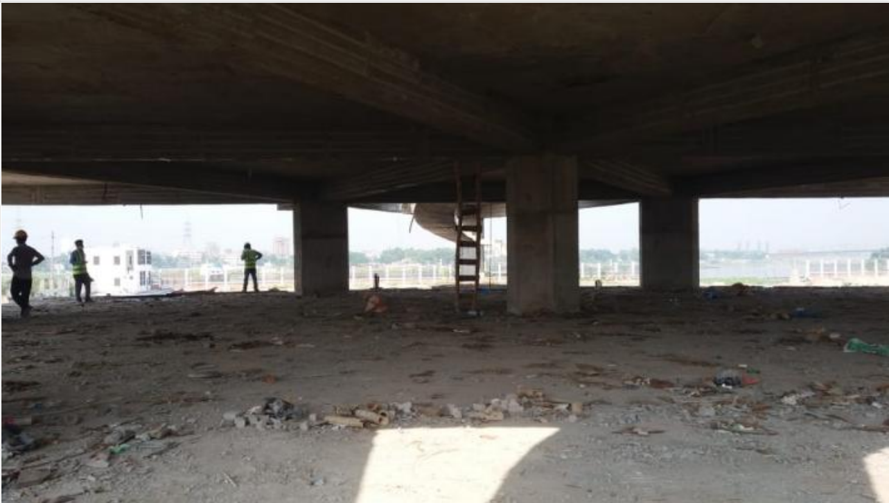
1st Floor Roof-De-shuttering on 25-04-21
