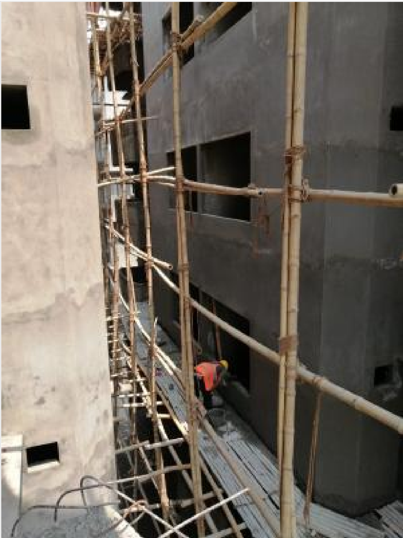
Out-side Plastering on 02-05-21
