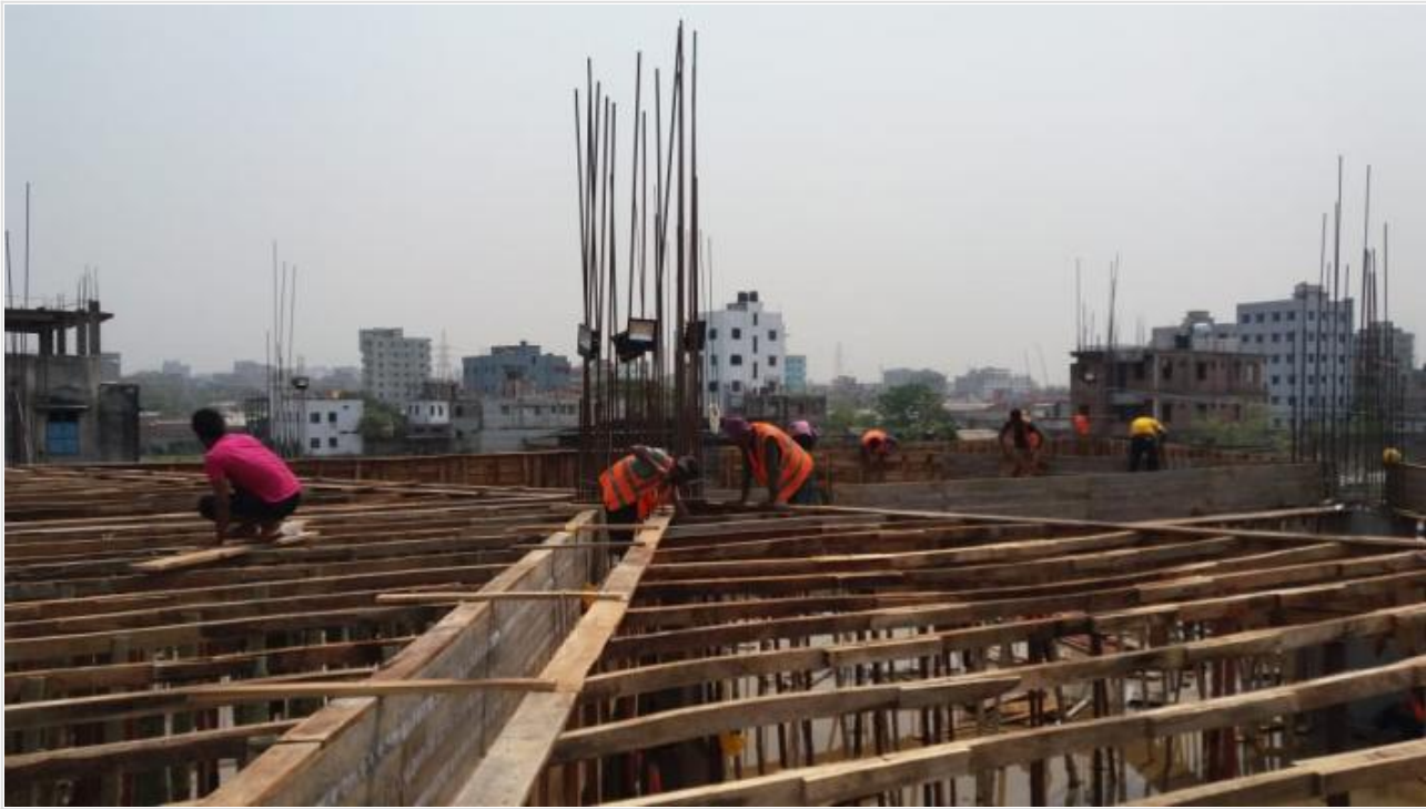
Mosque 1st Floor Slab Shuttering on 28-03-21
