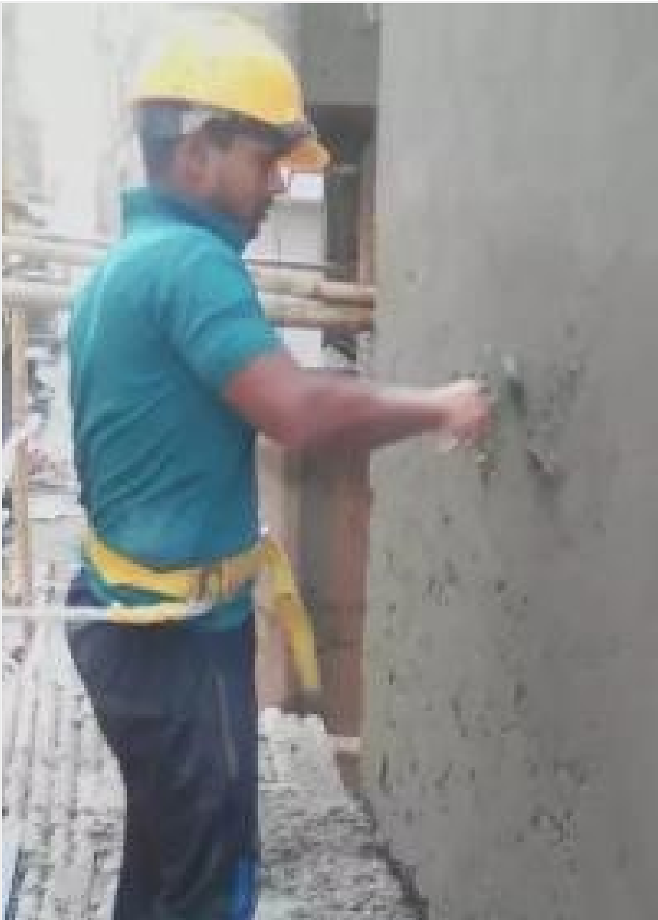
Out-side Plaster Work on 04-05-21
