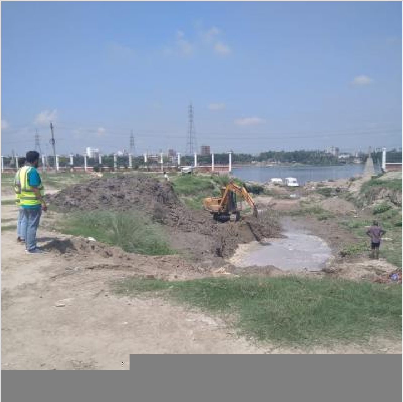
Landing Station-Excavation on 22-05-21
