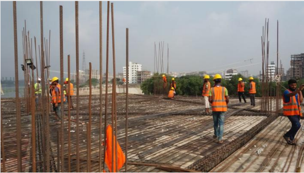
Mosque 1st Floor Slab Re-bar Work on 03-04-21
