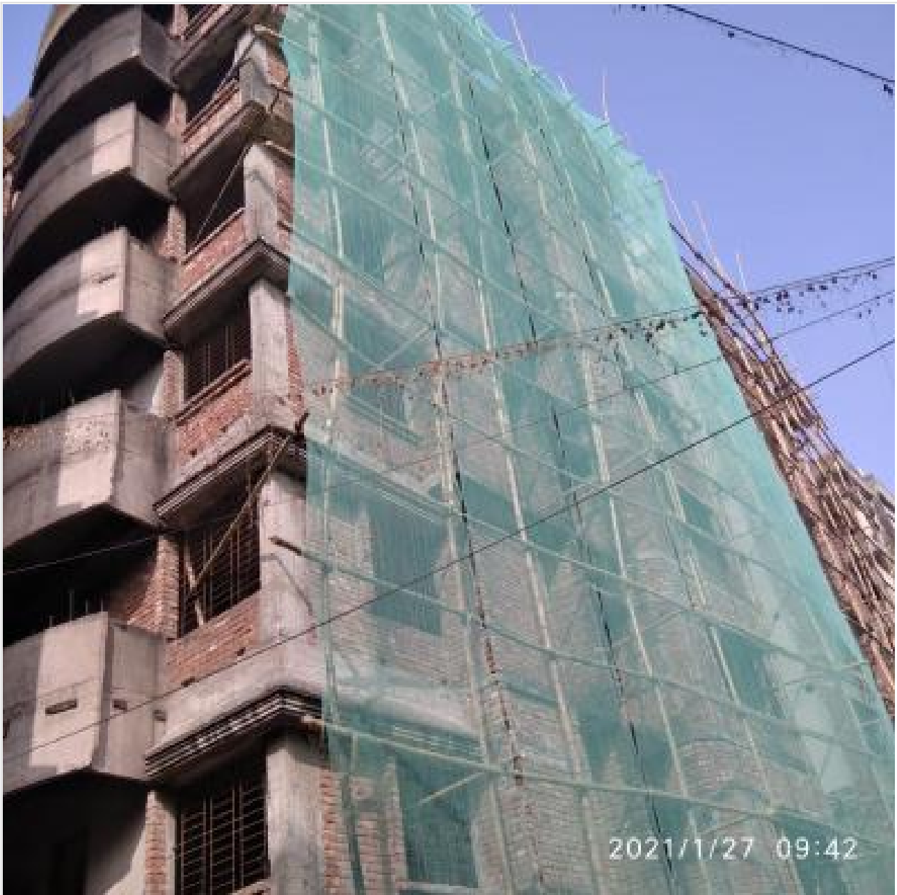
Scaffolding for Outside Plaster-Buildin on 27-01-21
