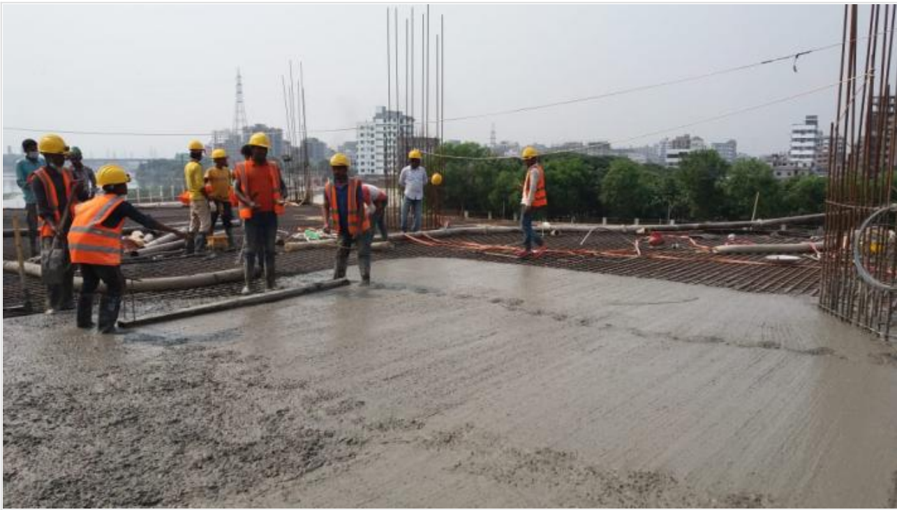
Mosque 1st Floor Slab Concreting on 06-04-21
