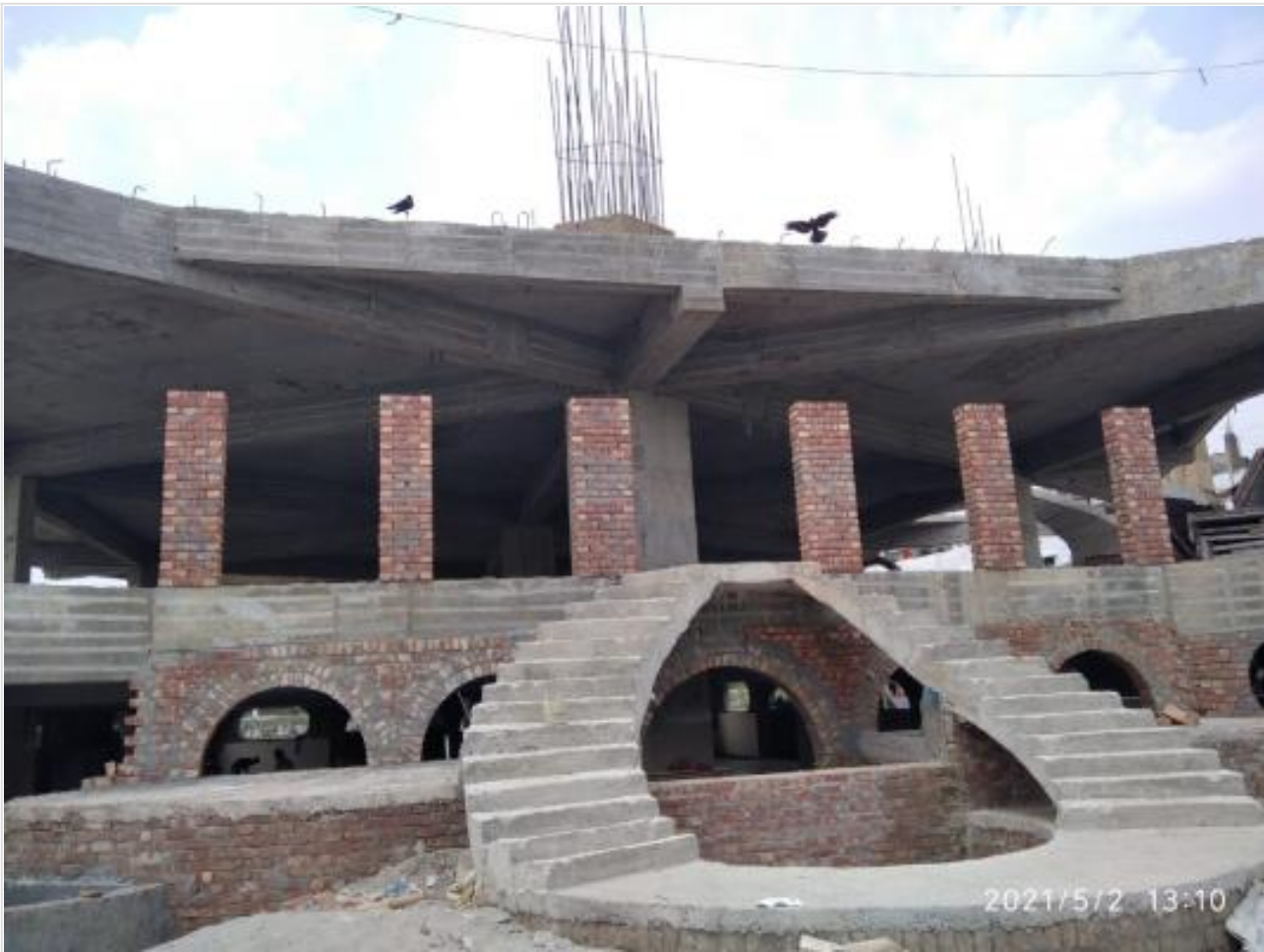
Mosque-Gr./1st Floor-Ancillary Works on 02-05-21
