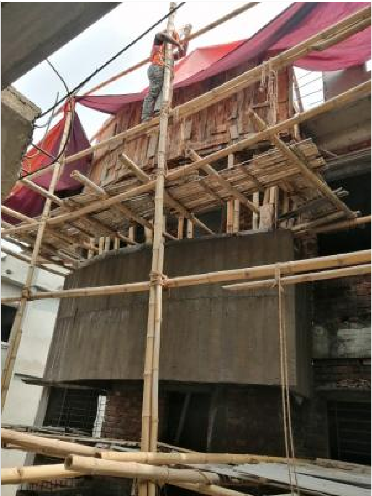
Drop Wall Shuttering on 28-04-21
