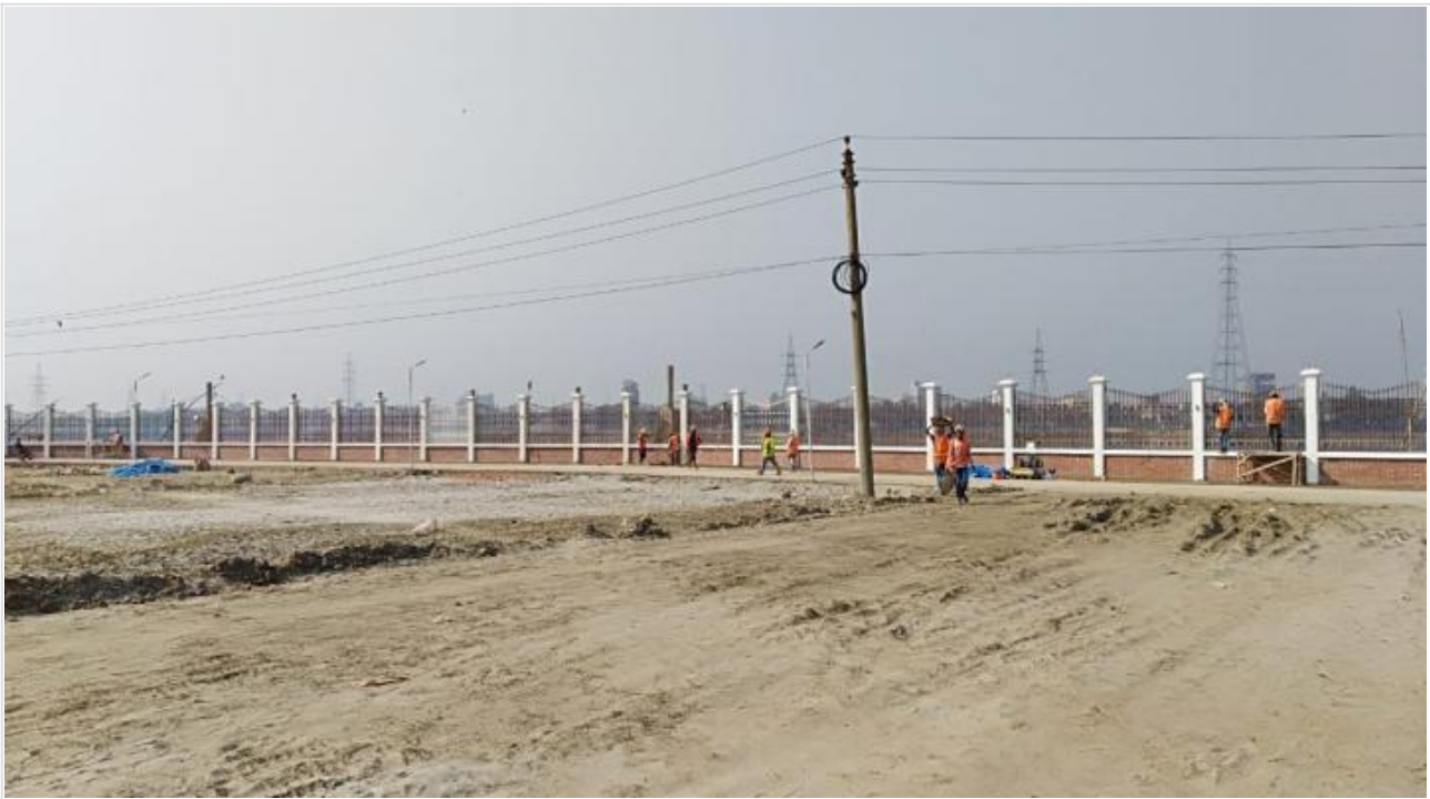
Riverside Boundary Fencing on 08-02-21
