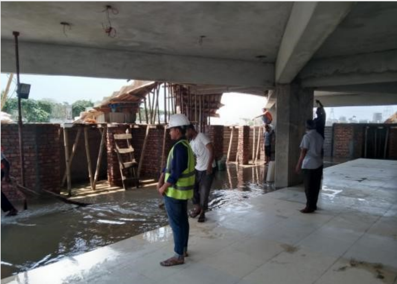
Mosque-Basement-Tile Work on 16-04-21
