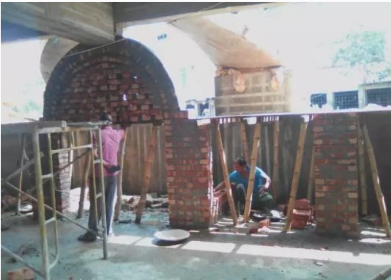
Mosque-Ground Floor Ancillary Works on 14-04-21
