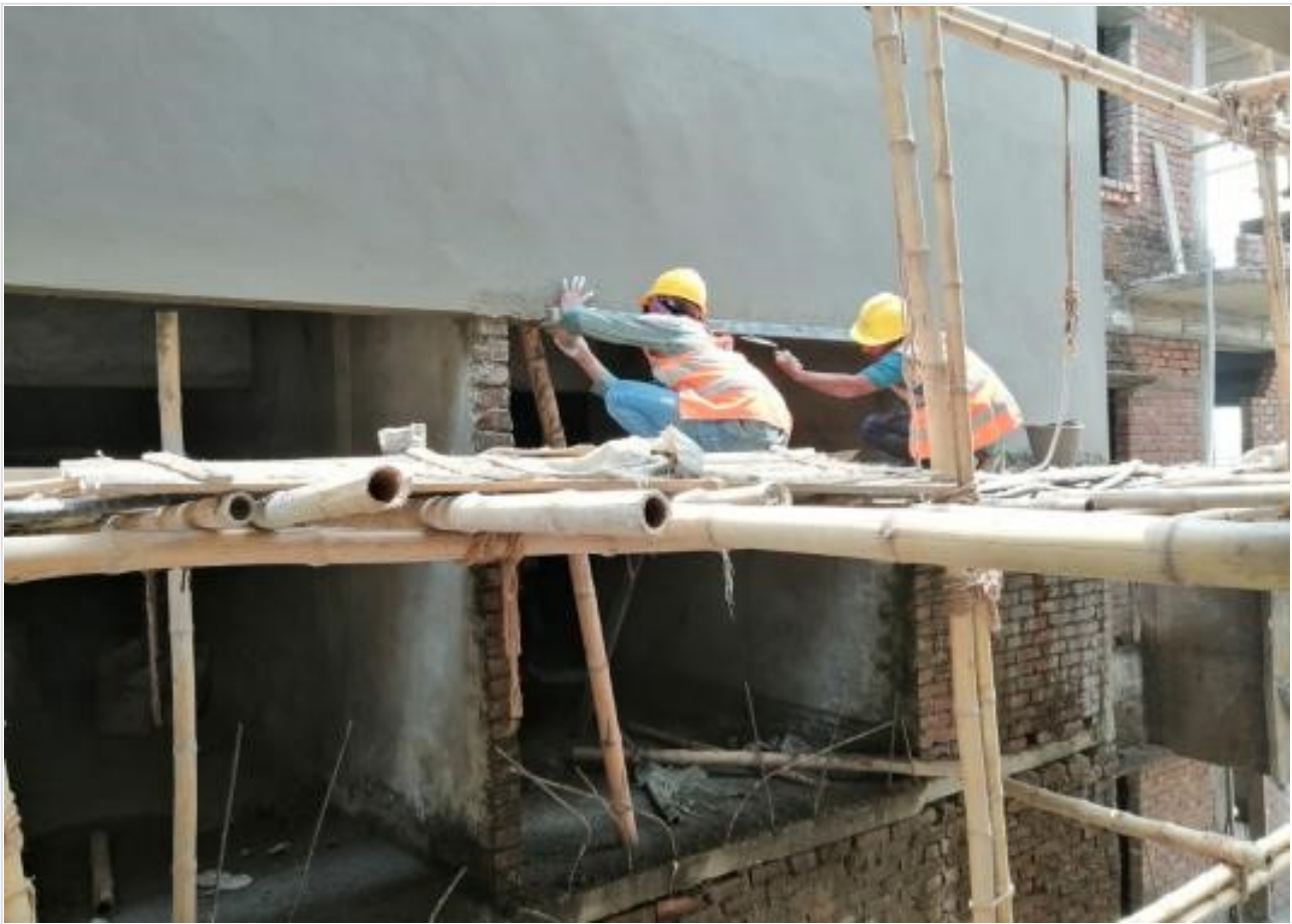
Out-side Plastering on 28-04-21
