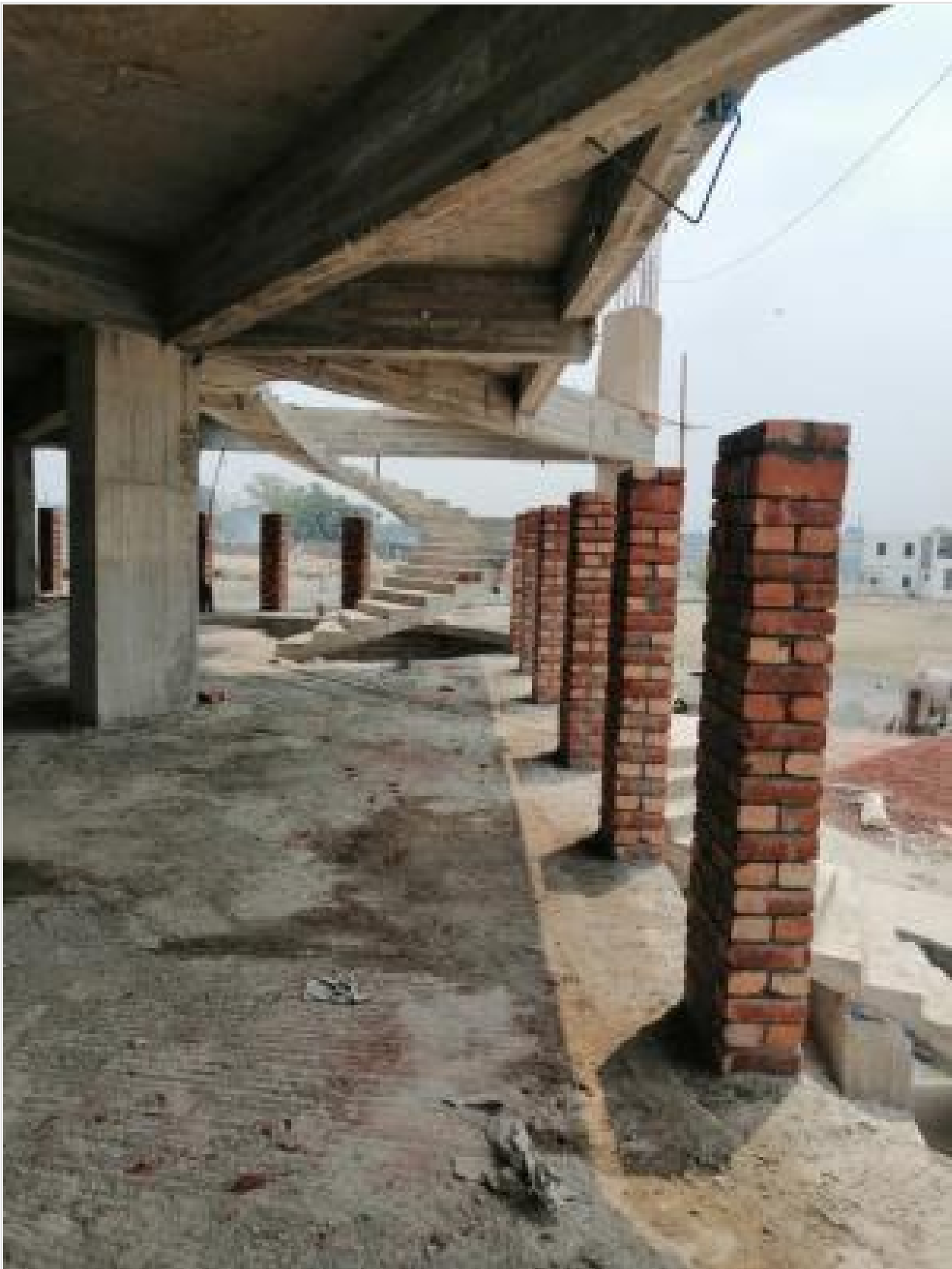
Out-side Plaster Work on 01-05-21
