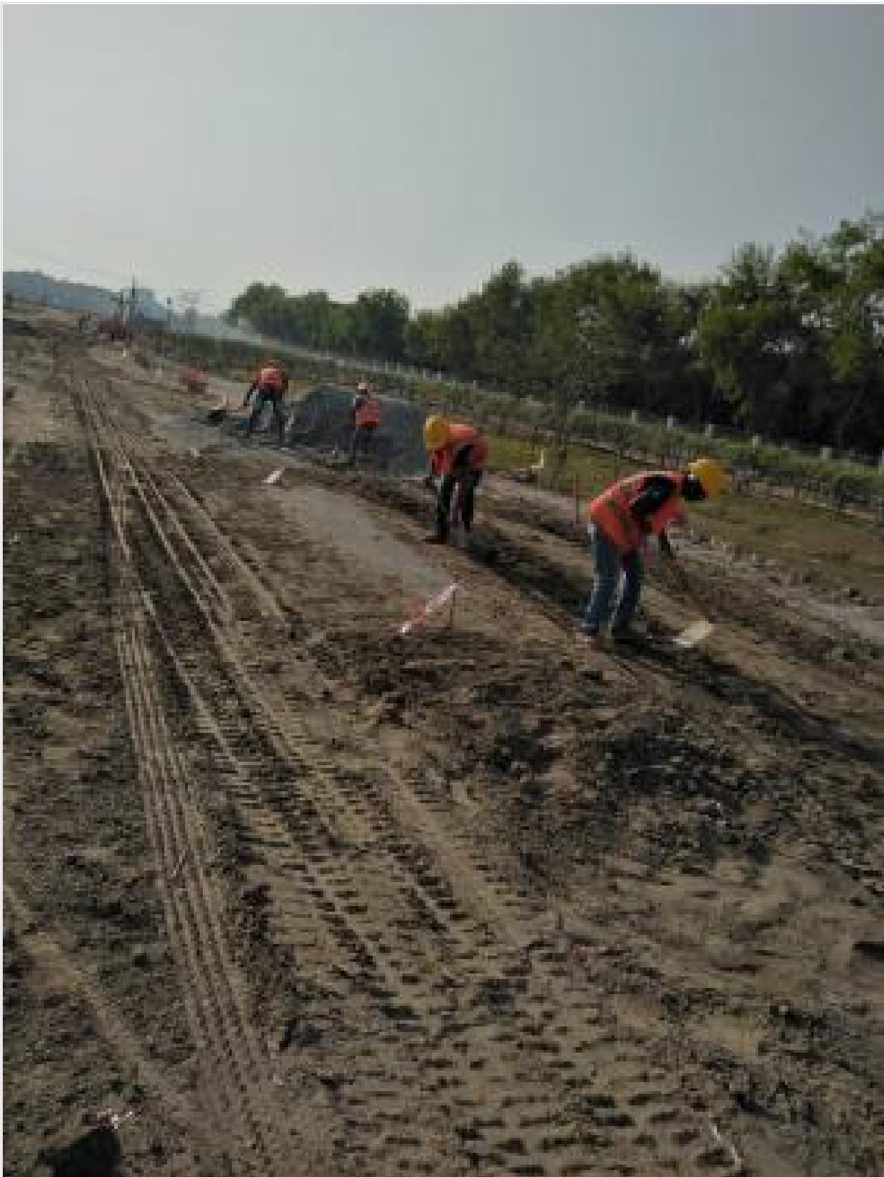
40 ft Road Levelling and dressing on 10-02-21
