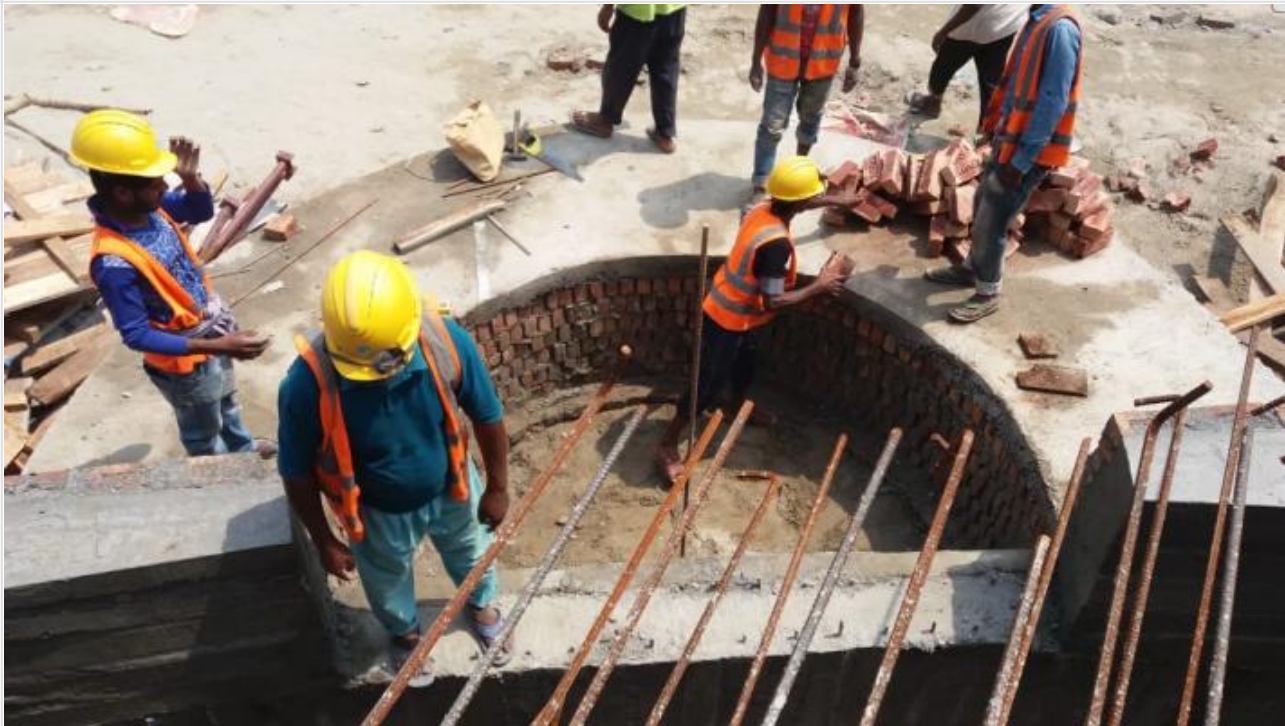
Mosque Ground Floor Stair Concreting on 28-03-21
