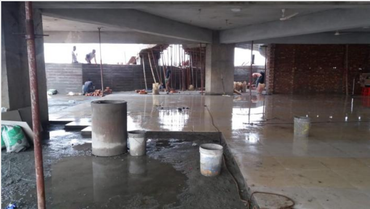
Mosque-Basement-Tile Work on 13-04-21
