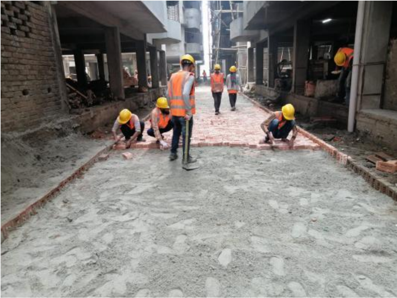
Inner Road CC Work on 27-01-21
