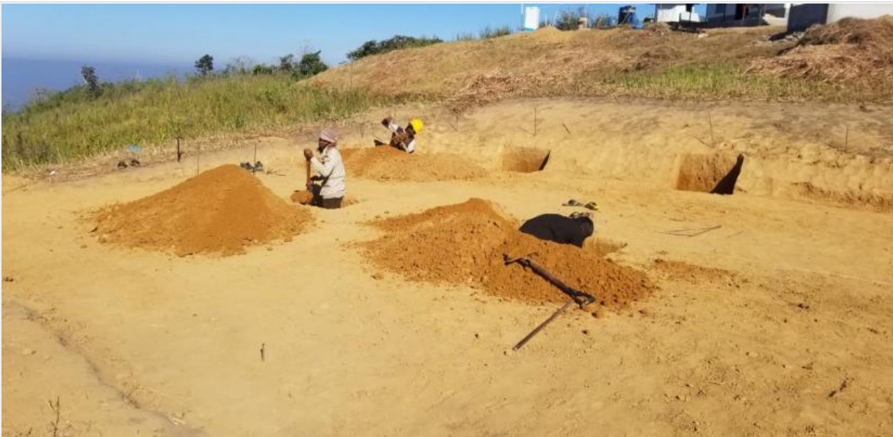
Guest House-Excavation on 09-01-21
