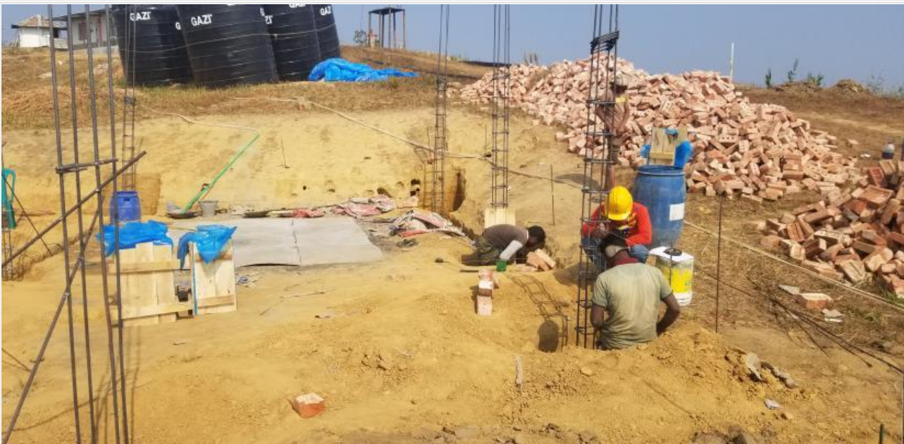
Shuttering fitting work for short column on 16-01-21
