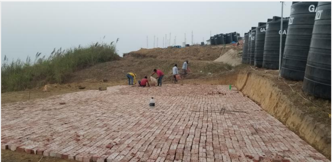
Brick soling work for water tank placei on 19-01-21
