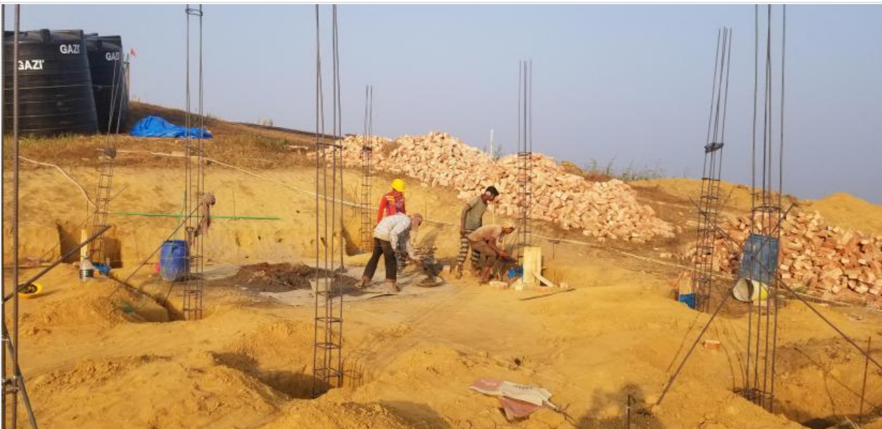
Short column casting work for guest hous on 16-01-21
