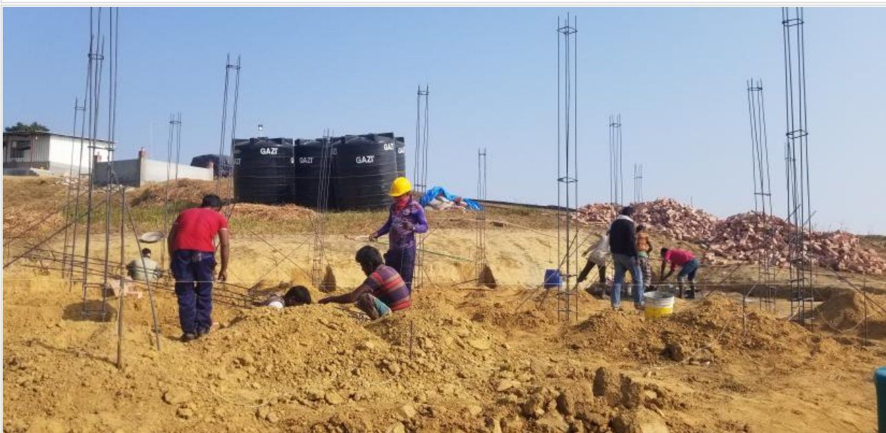
Column standing work on going at G.House on 15-01-21
