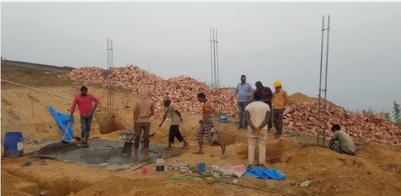
Footing & column casting work on going on 13-01-21
