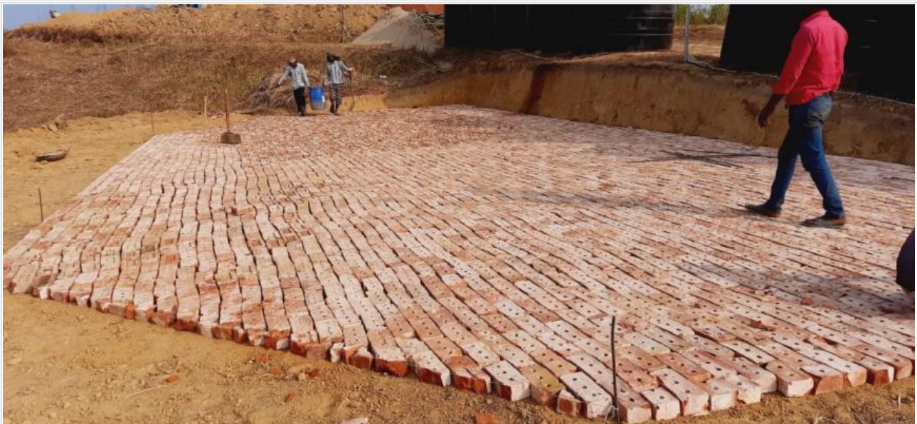
Soling for PVC Water Tank on 20-01-21
