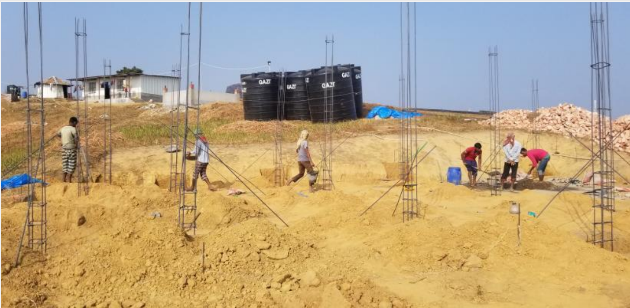
Footing casting work on going at G.House on 15-01-21
