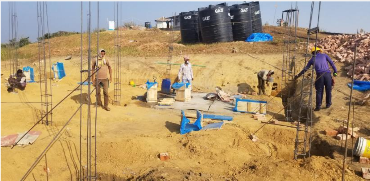
Shuttering fitting work for short column on 17-01-21
