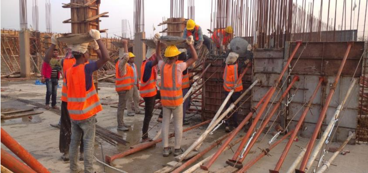
Retaining wall and Column Concreting on 28-01-21
