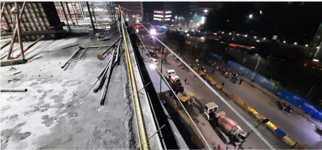
Night Shift Working on 16-01-21
