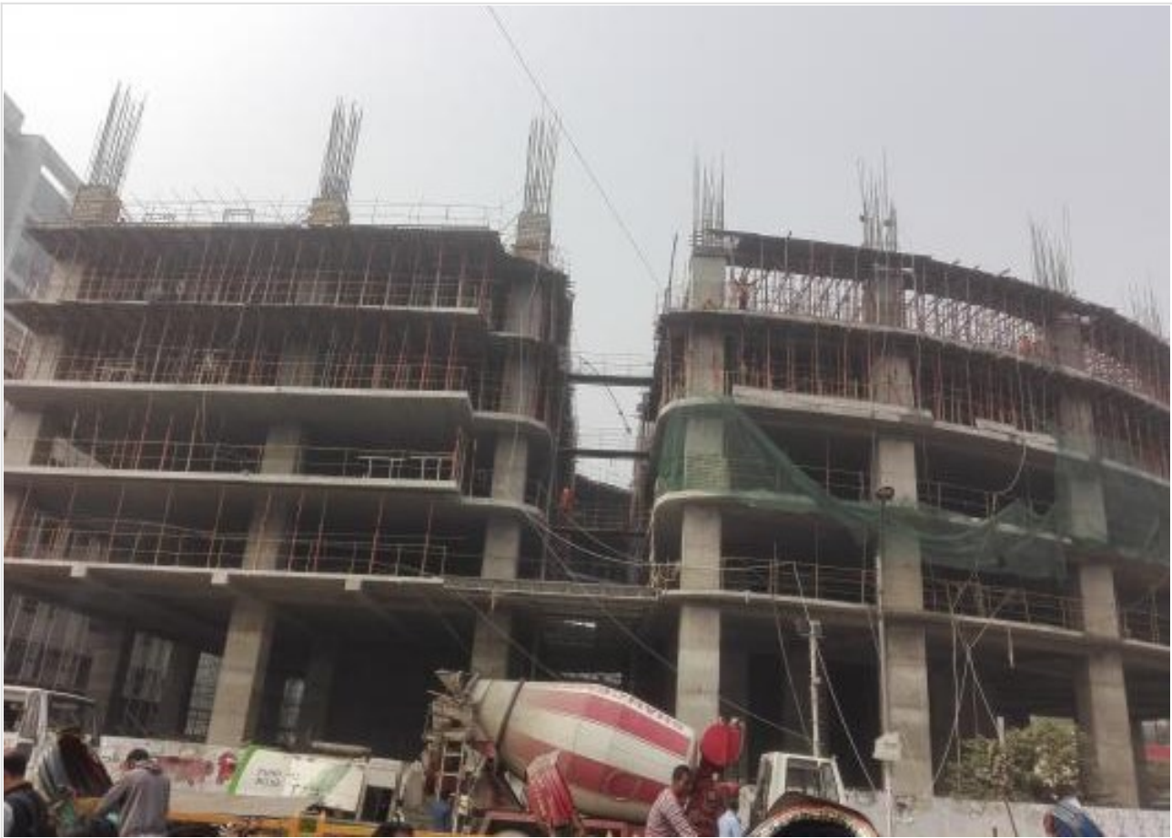
Project Picture on 24-01-21
