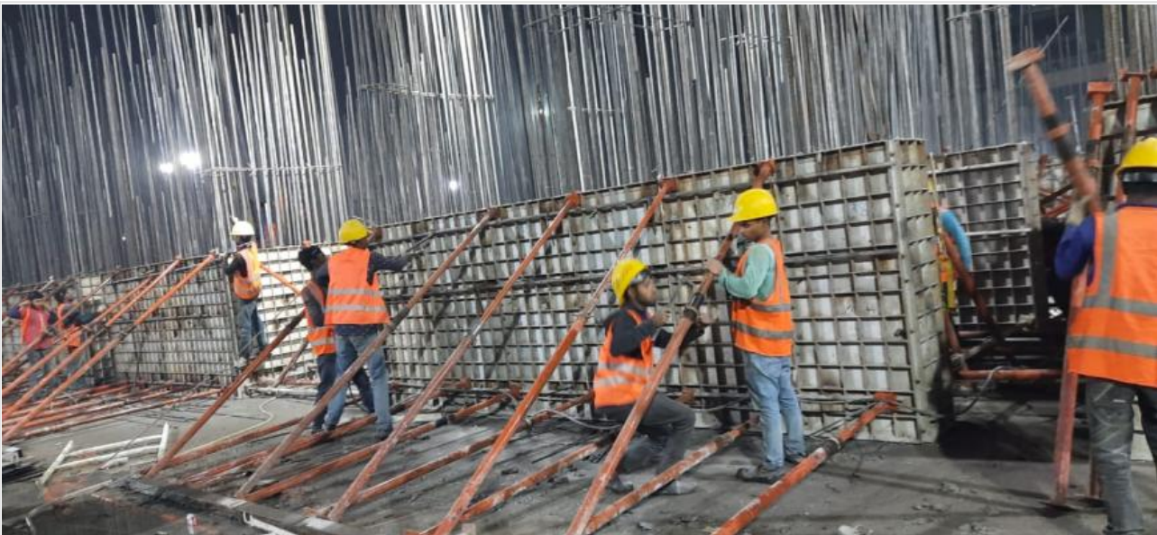
Lift Core Wall Shoring on 14-01-21
