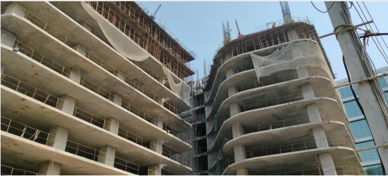
8th Floor North Tower Roof Slab Casting on 05-04-21
