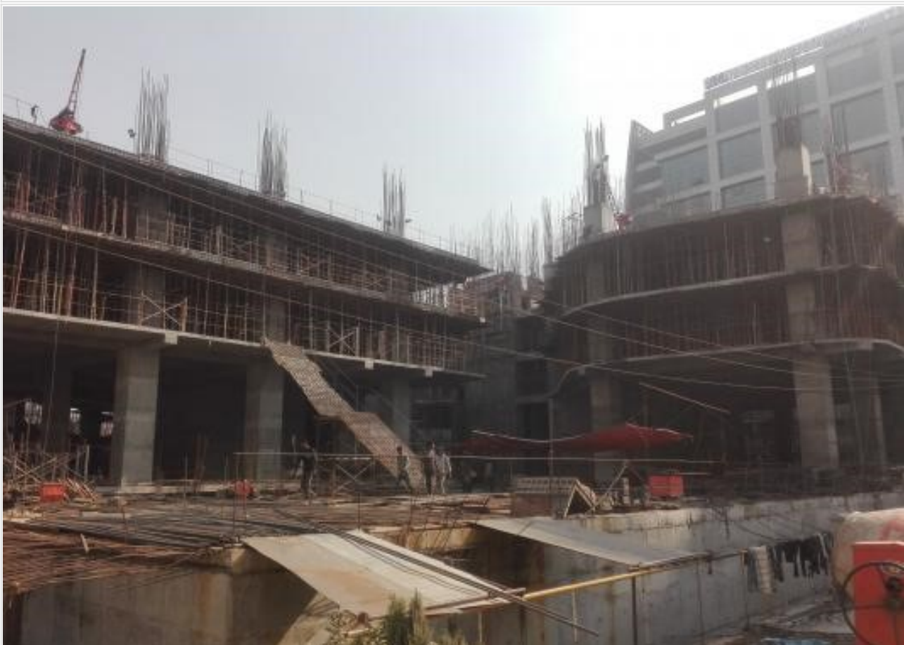
3rd Floor South Tower-Stair Complete on 11-01-21
