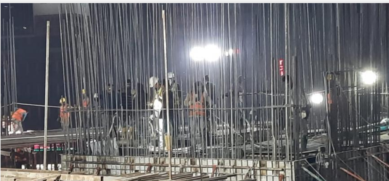
Re-bar Work on 18-01-21
