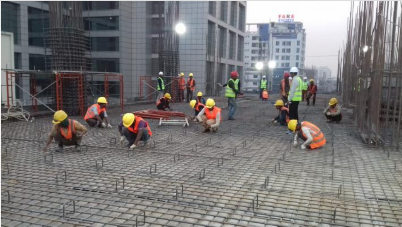
Slab Re-bar Work on 30-01-21
