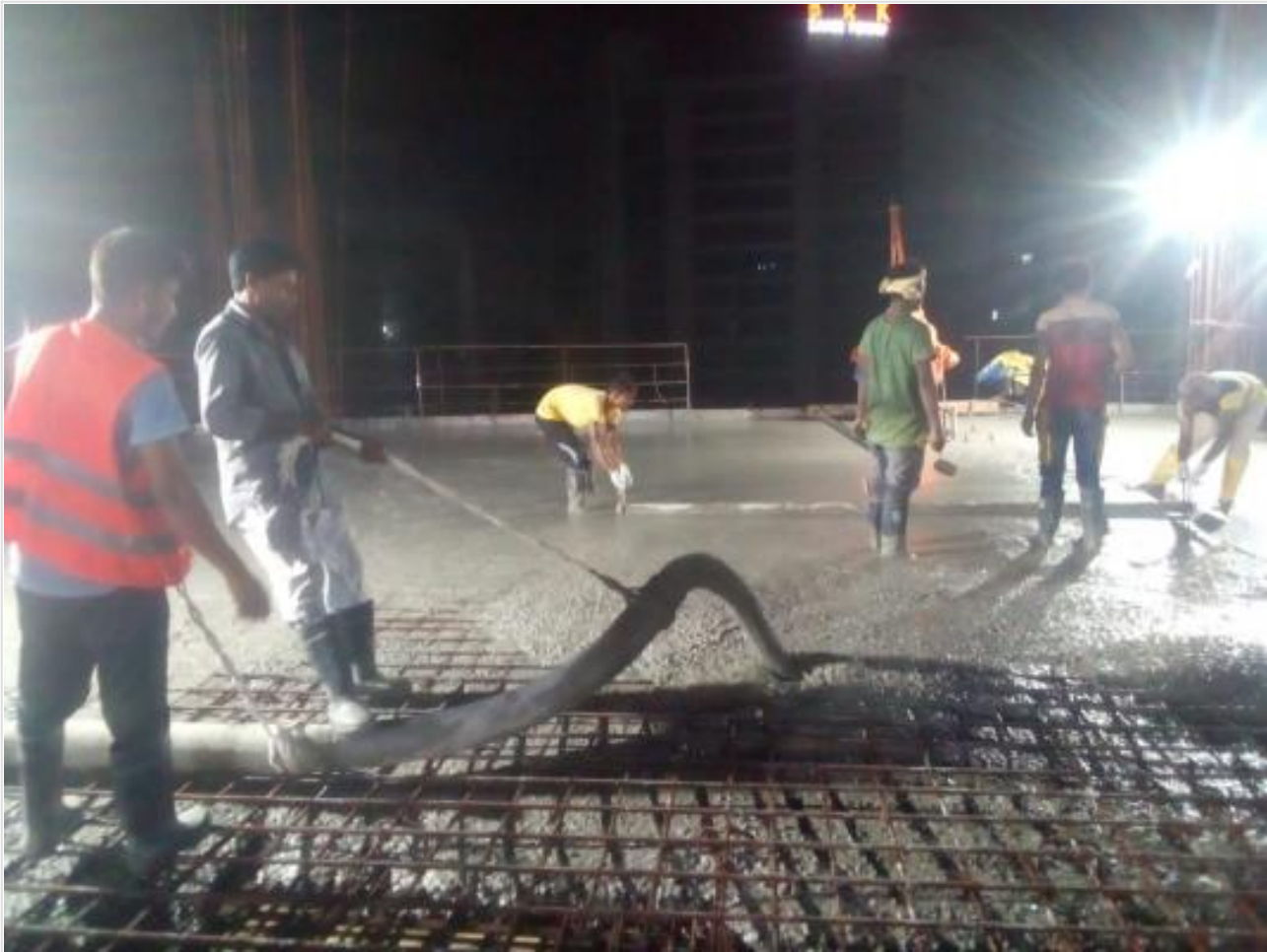
South Tower 11th Floor Slab Concreting on 02-09-21
