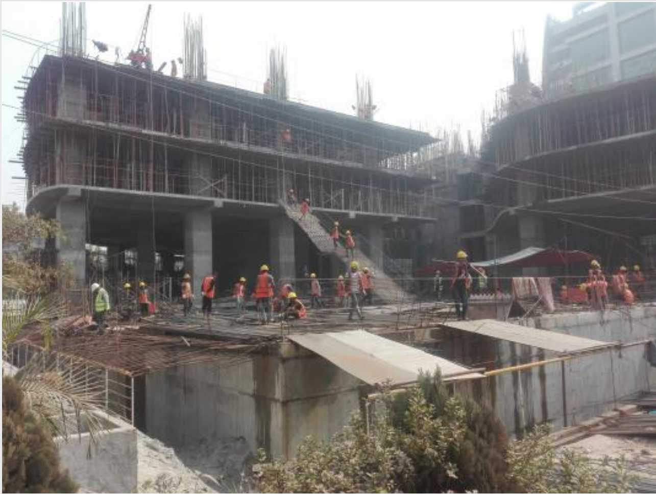
3rd Floor South Tower-Column Complete on 06-01-21
