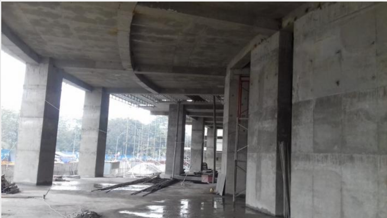
Inside Building on 29-01-21
