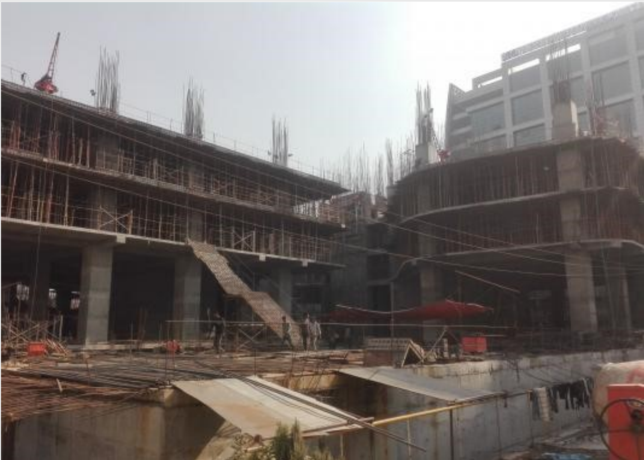
3rd Floor South Tower Slab Complete on 11-01-21
