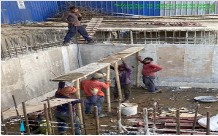
Tank slab shuttering on 19-11-24
