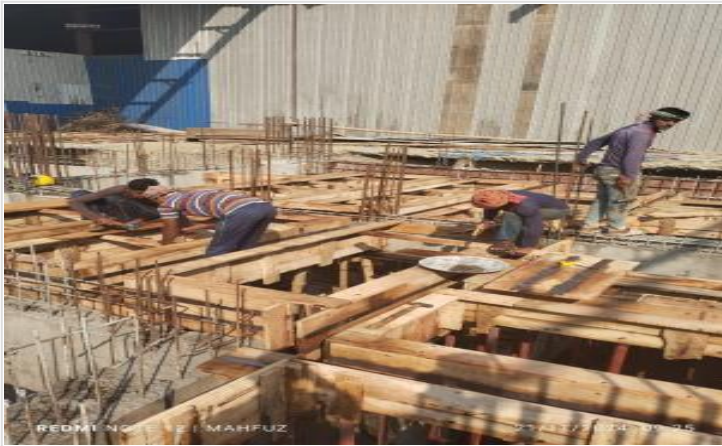
Tank slab shuttering on 22-11-24
