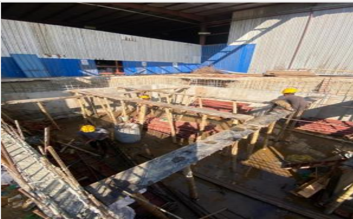
Tank slab shuttering on 20-11-24
