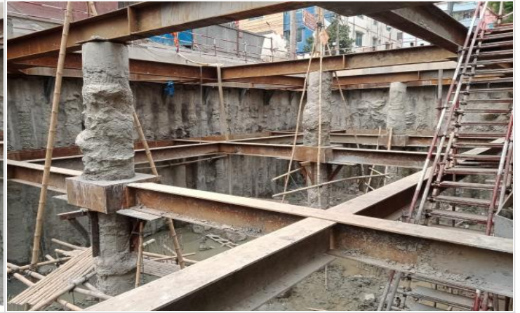
Pile gap water proofing on 30-04-22
