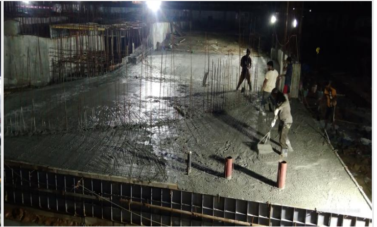
Ready mix concreting on 03-06-22
