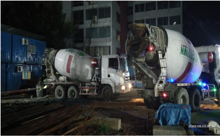
Ready mix car on 03-06-22
