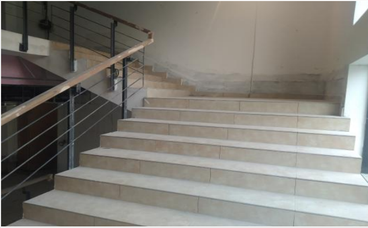
Tiles work on 31-01-22
