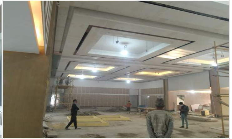
Interior work on 31-01-22
