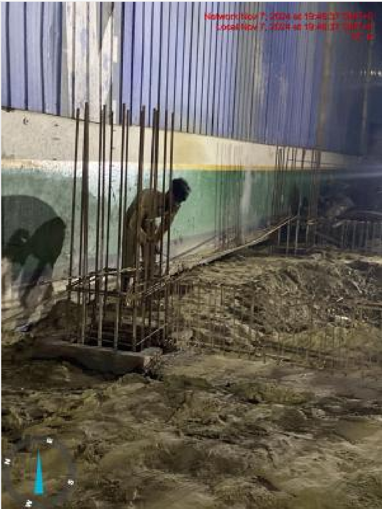
Column re-bar work on 07-11-24
