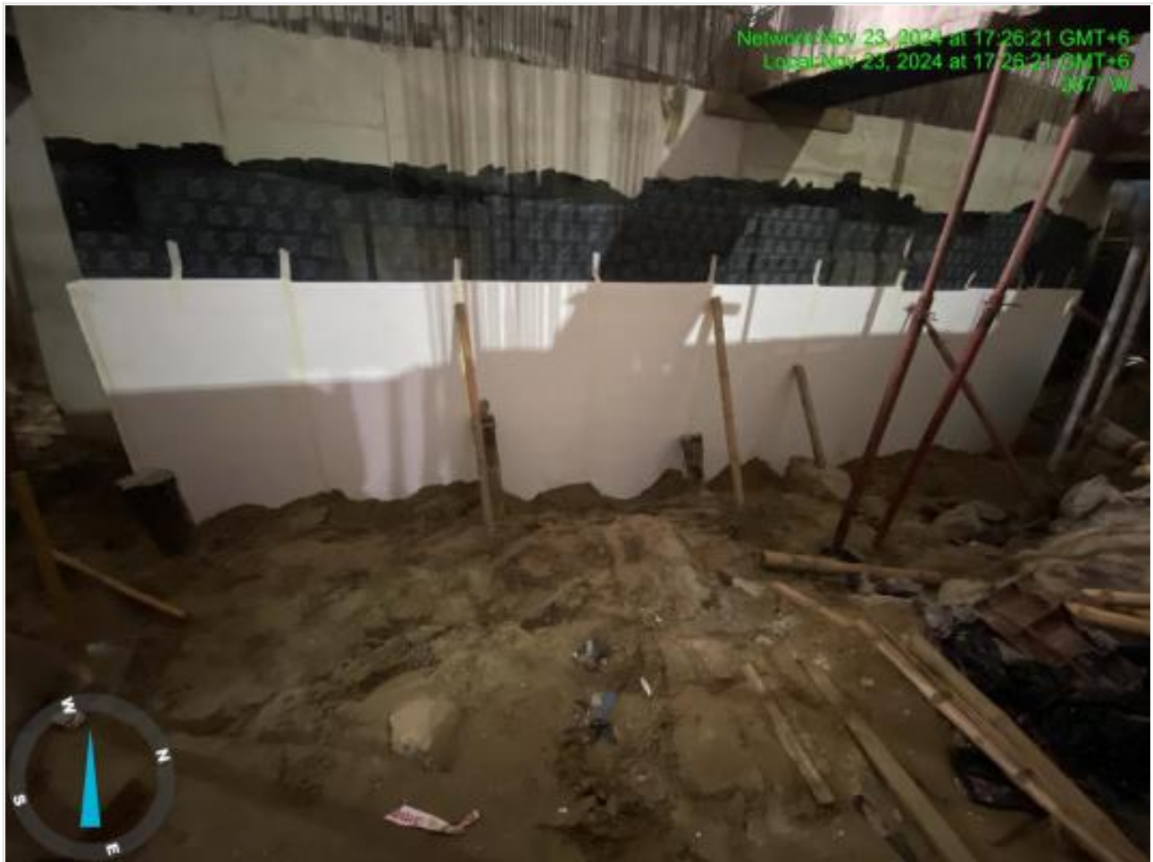
Tank wall stylo foam fixing on 23-11-24
