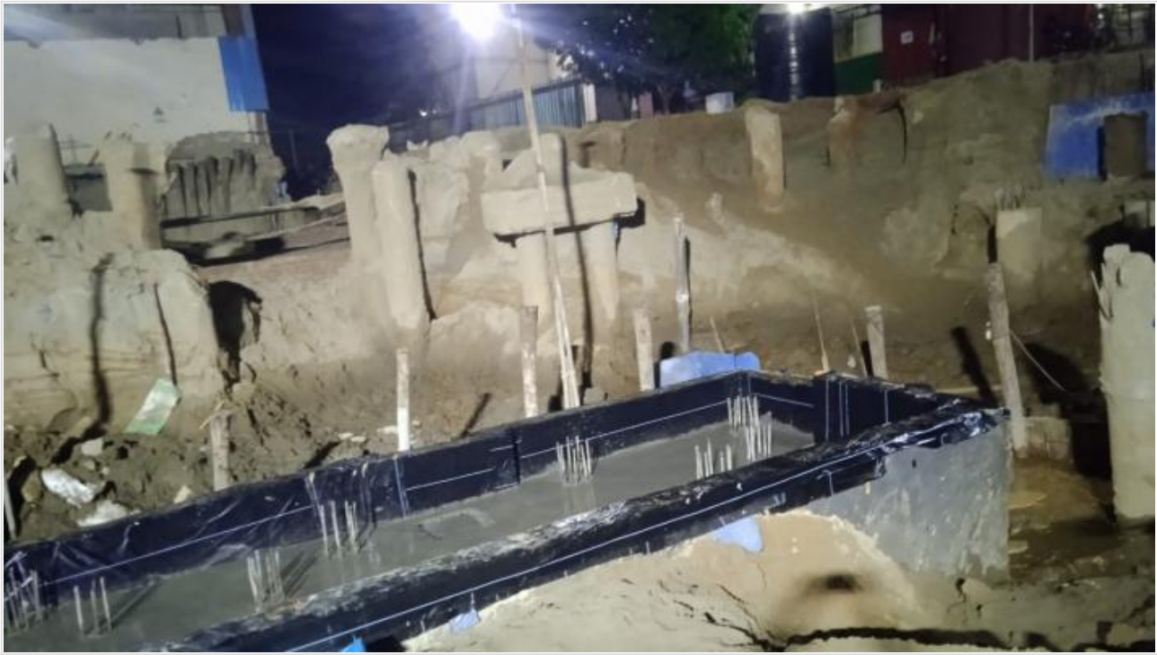
Tank base top mortering on 22-10-24
