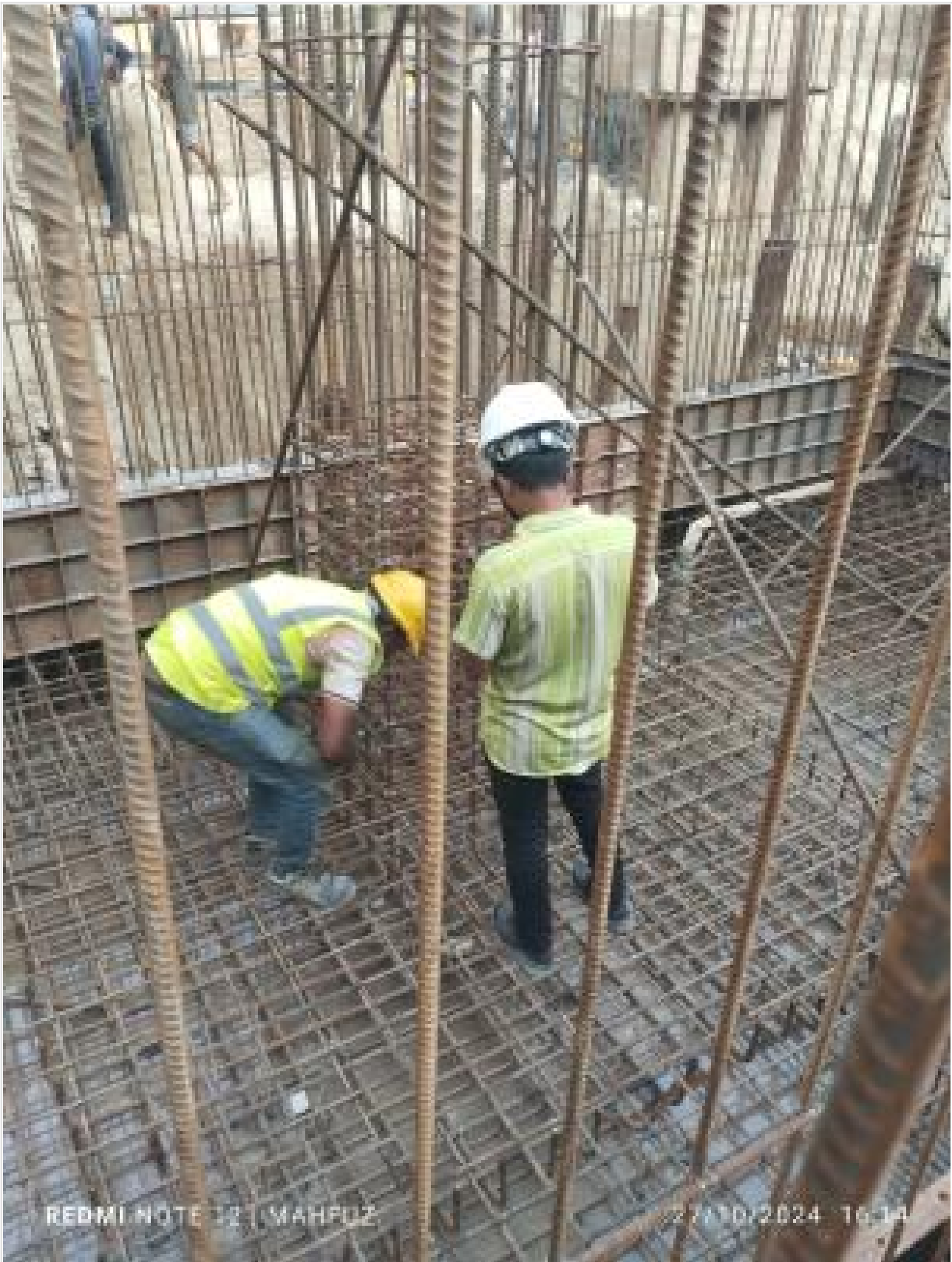
Tank wall shuttering on 27-10-24
