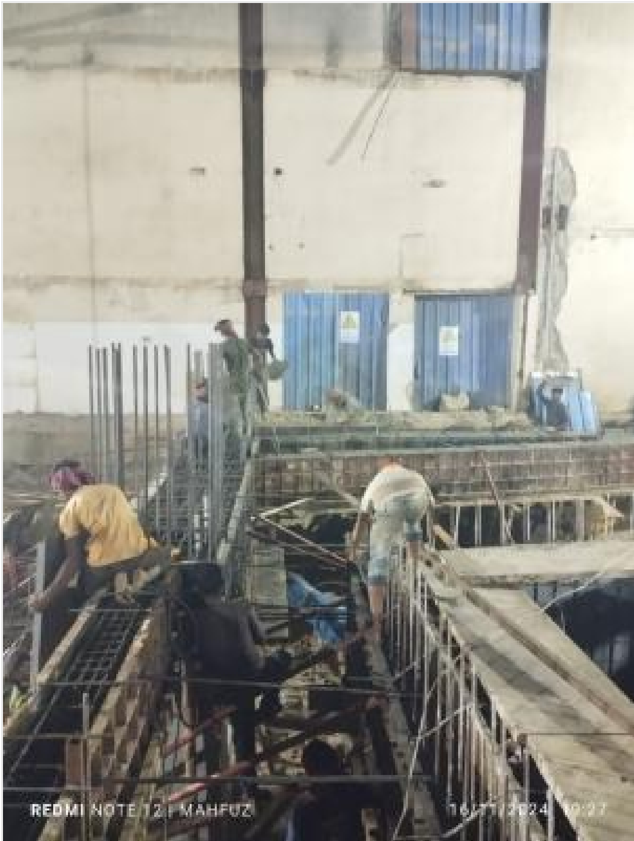
Foundation beam concreting on 16-11-24
