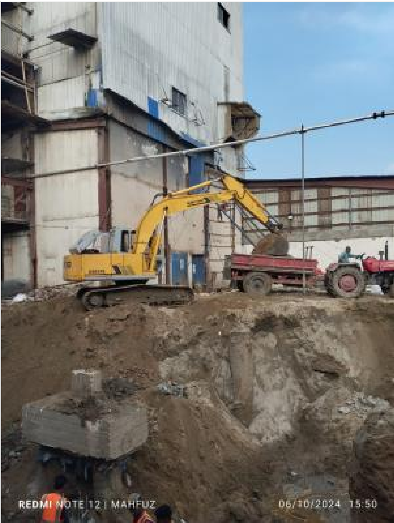
Earth Excavation on 06-10-24
