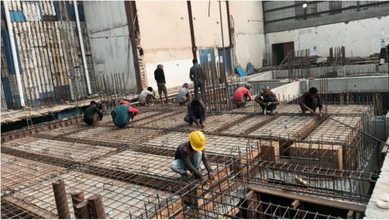
Tank slab re-bar work on 24-11-24
