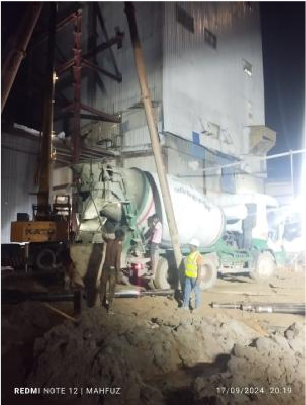
Pile concreting on 17-09-24
