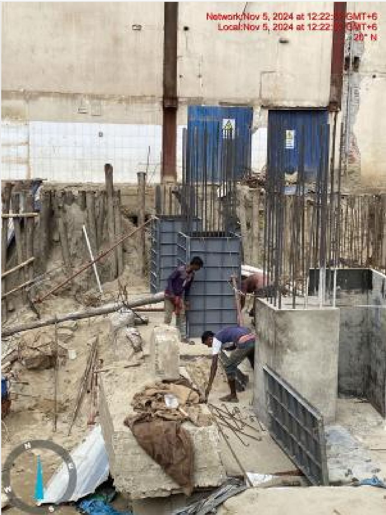
Column shuttering on 05-11-24
