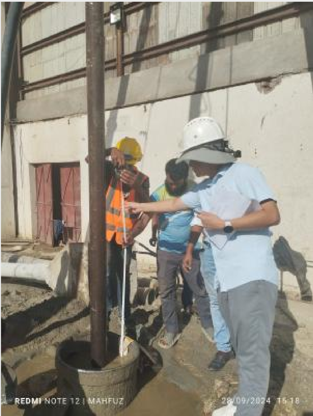
Pile boring depth checking on 28-09-24
