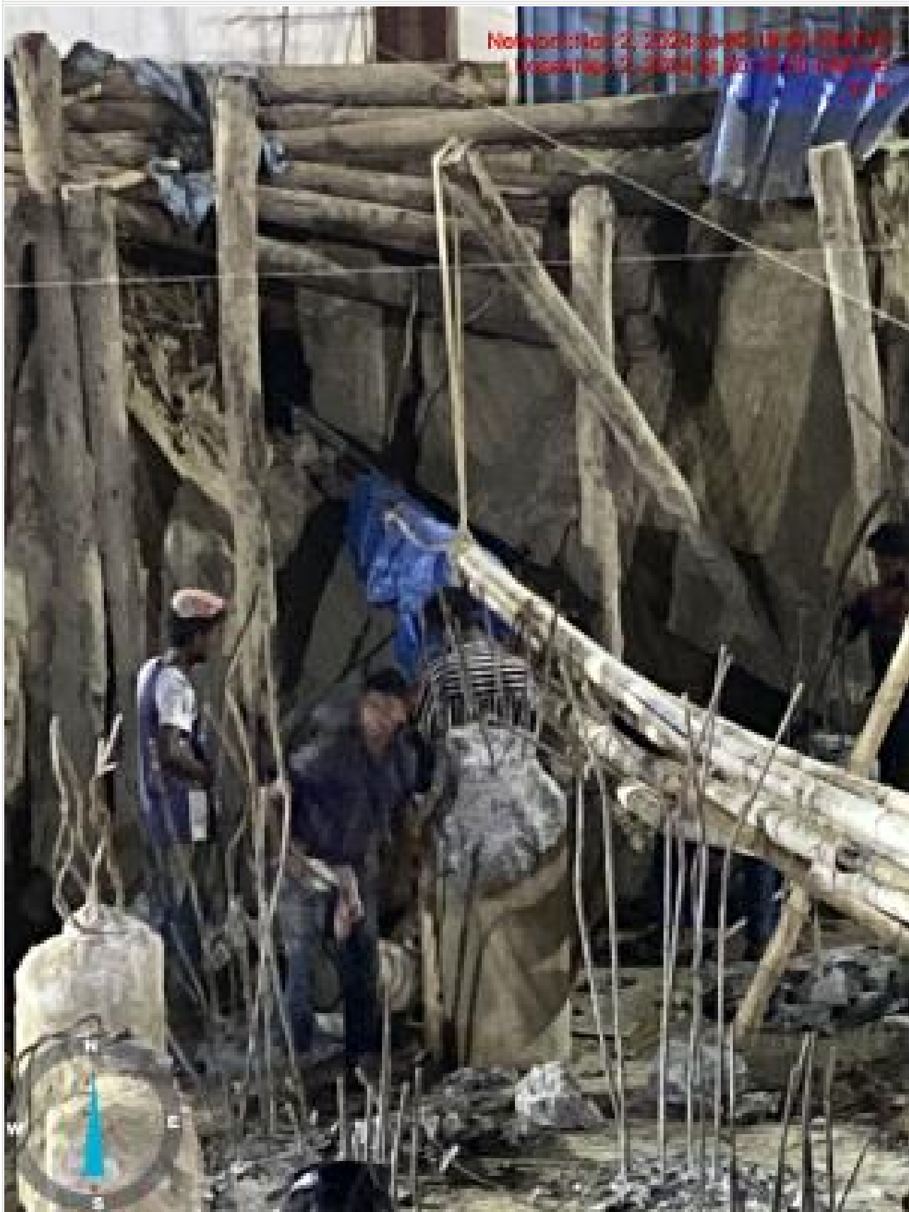
Pile head breaking on 02-11-24
