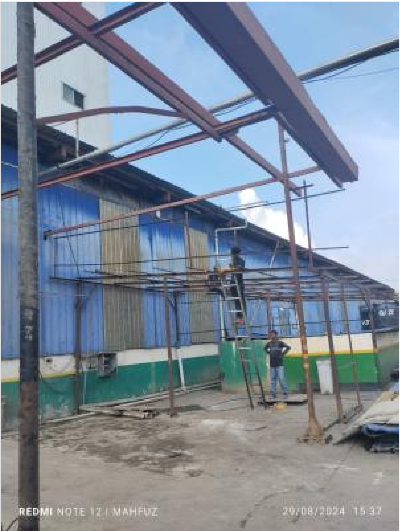
Sheet removing on 29-08-24
