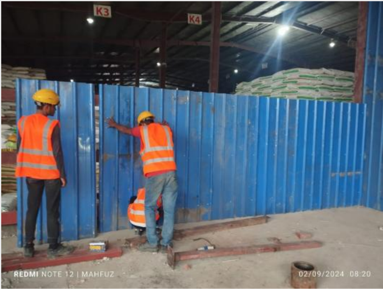
Fencing work on 02-09-24
