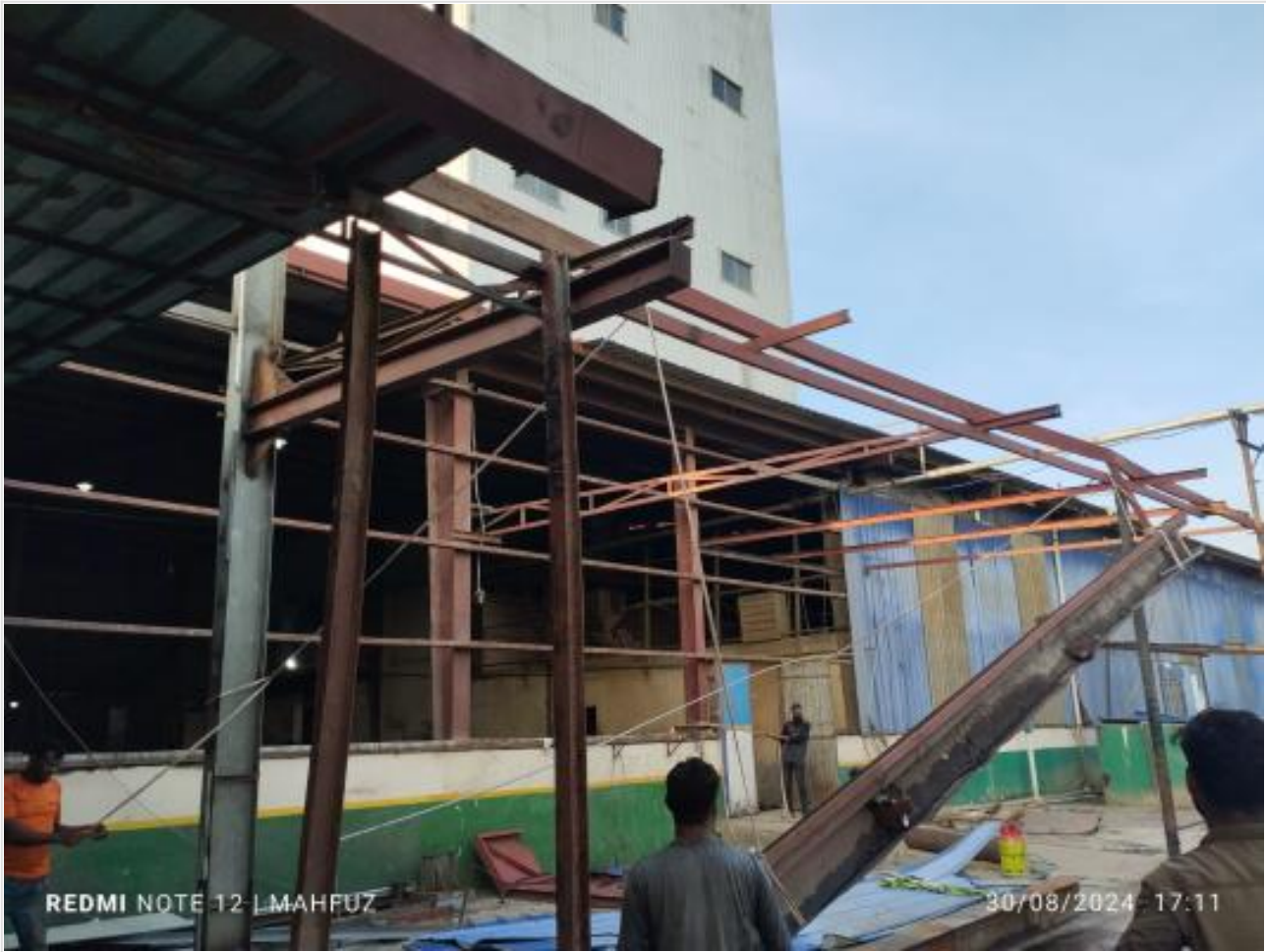
Steel beam removing on 30-08-24
