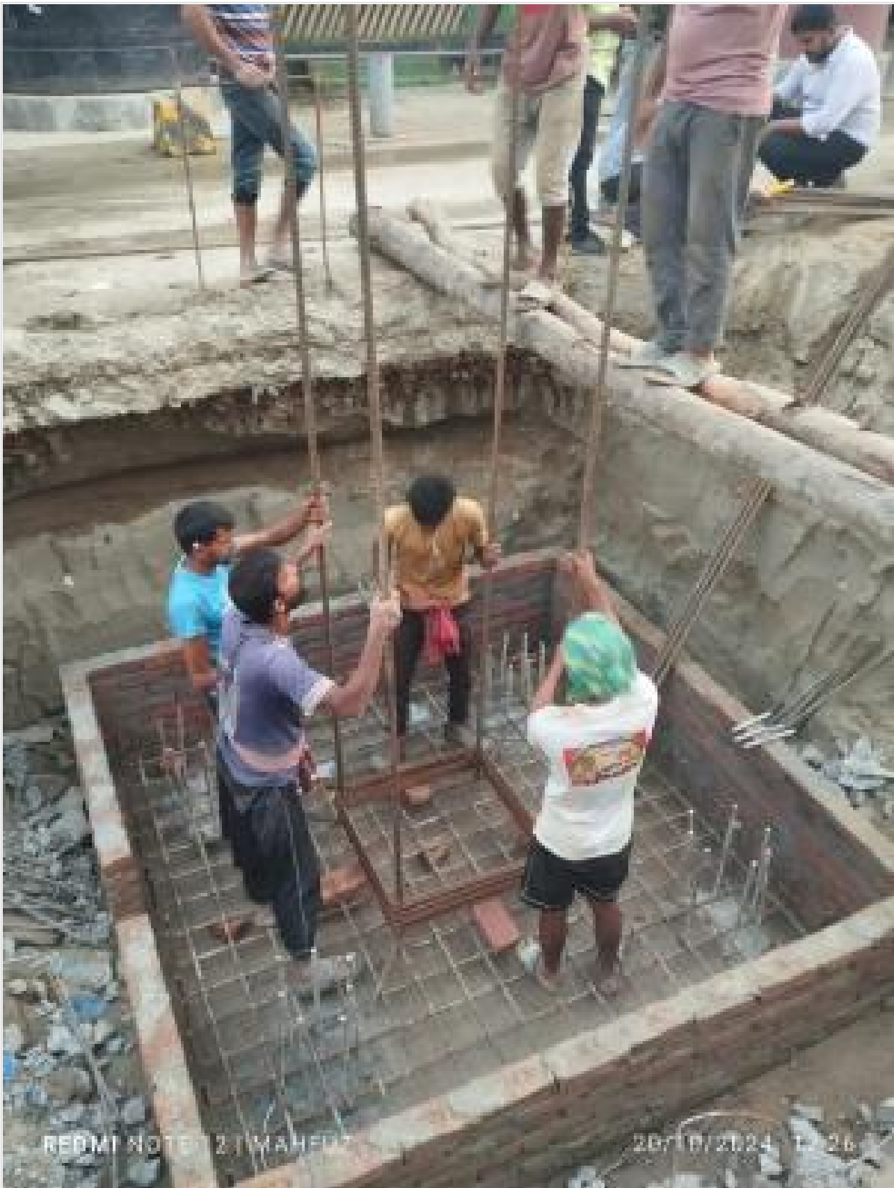
Pile cap re-bar work on 20-10-24
