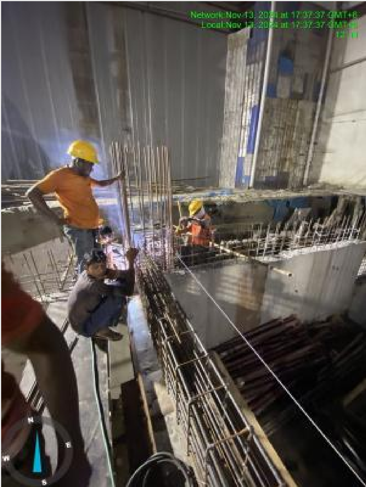
Foundation beam concreting on 13-11-24
