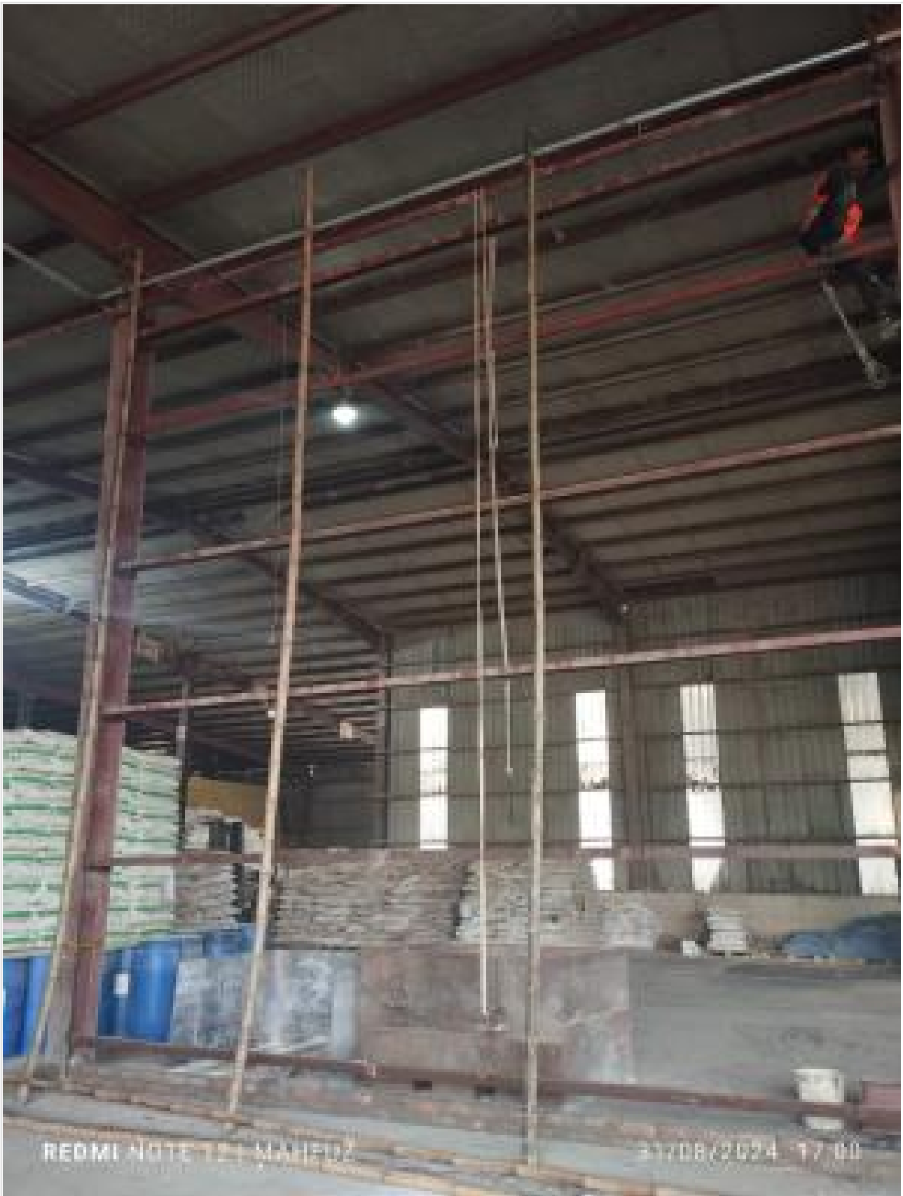
Fencing framing on 31-08-24
