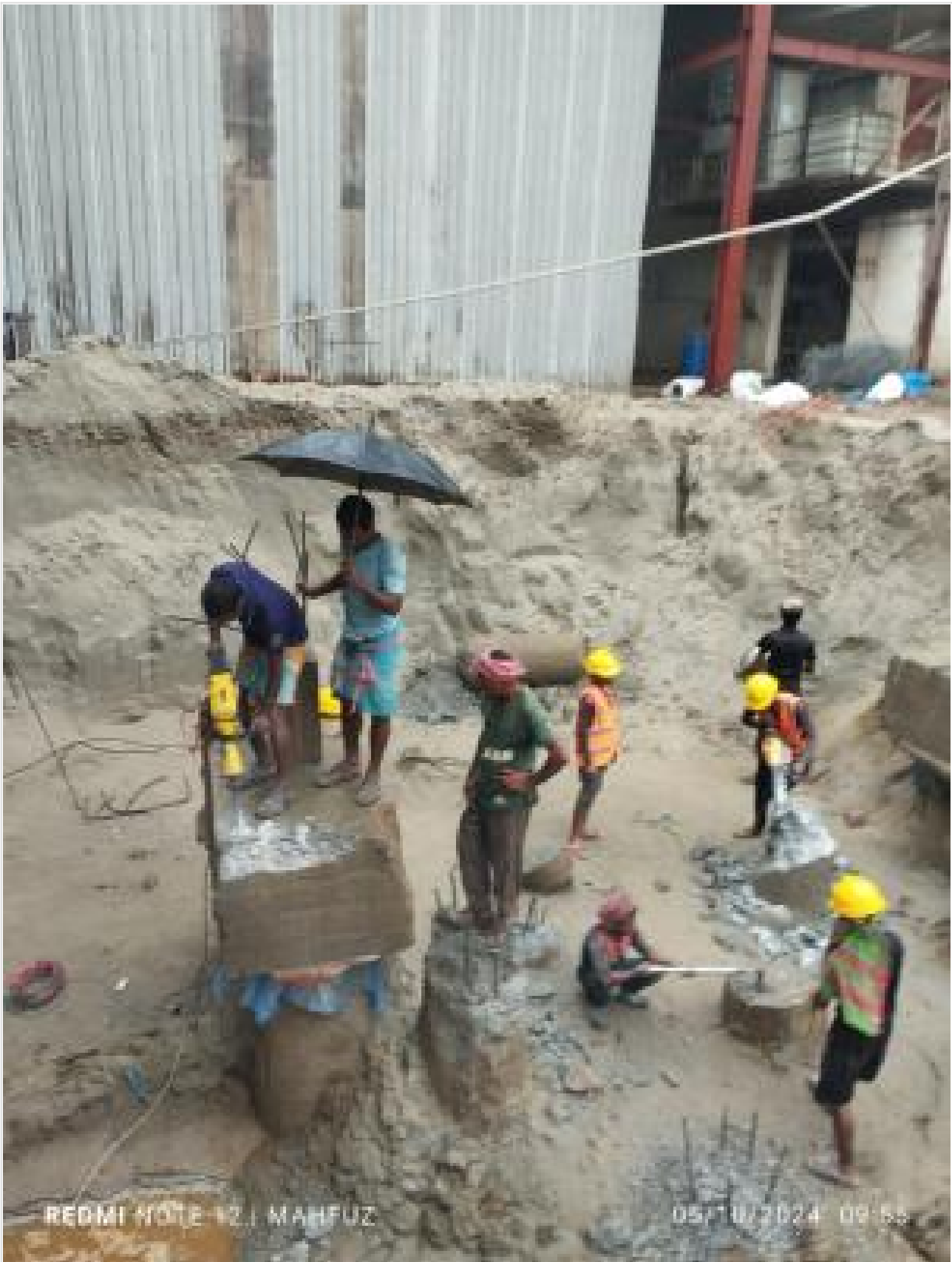
Old base breaking on 05-10-24
