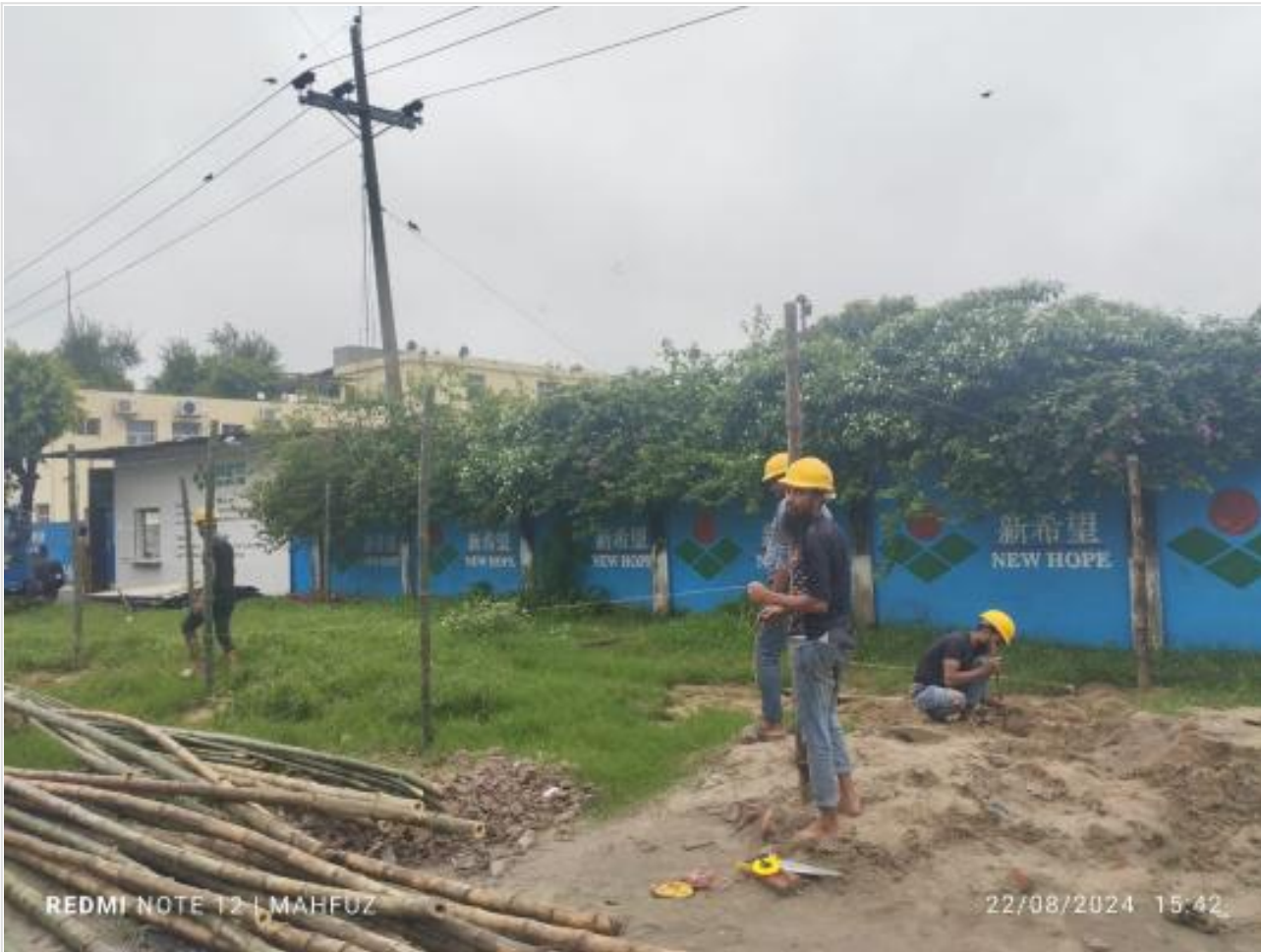
Labor Shed Making on 22-08-24
