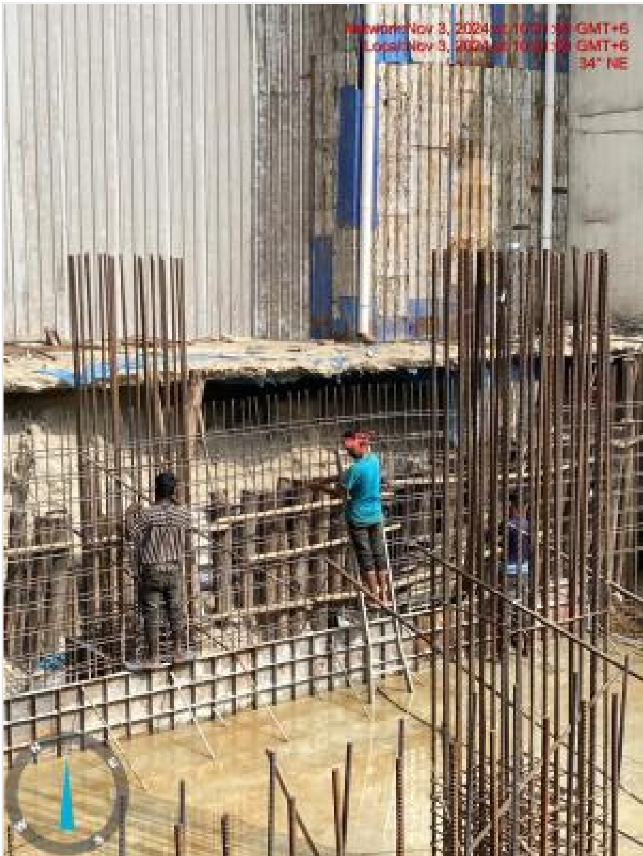
Wall re-bar work on 03-11-24
