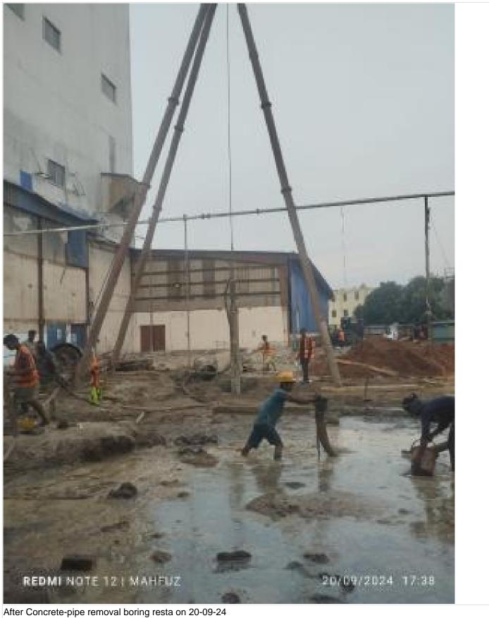
After Concrete-pipe removal boring resta on 20-09 During boring pile no.35 grid-2B Old concrete-MS pipe found
