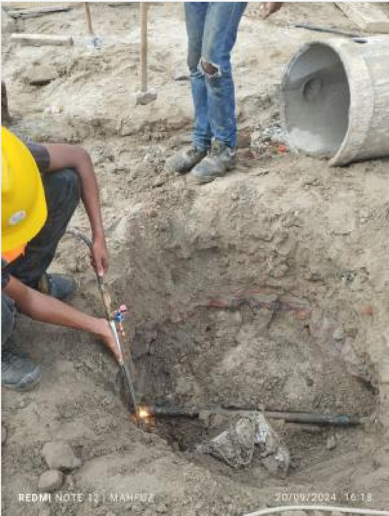
During boring old concrete-pipe found on 20-09-24
