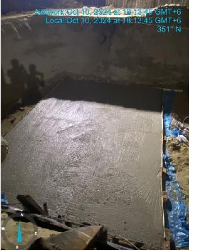
Water Reservoir Base CC-Bottom on 10-10-24 Old base dismantling 4 m3 by hydraulic hammer
