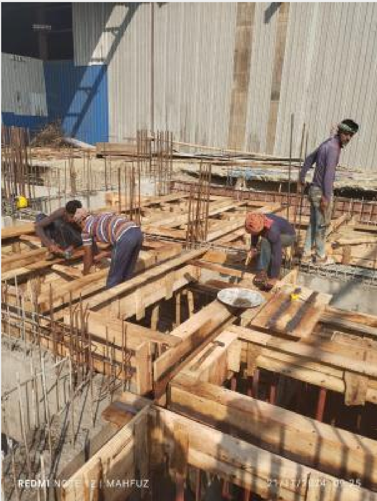
Tank slab shuttering on 22-11-24
