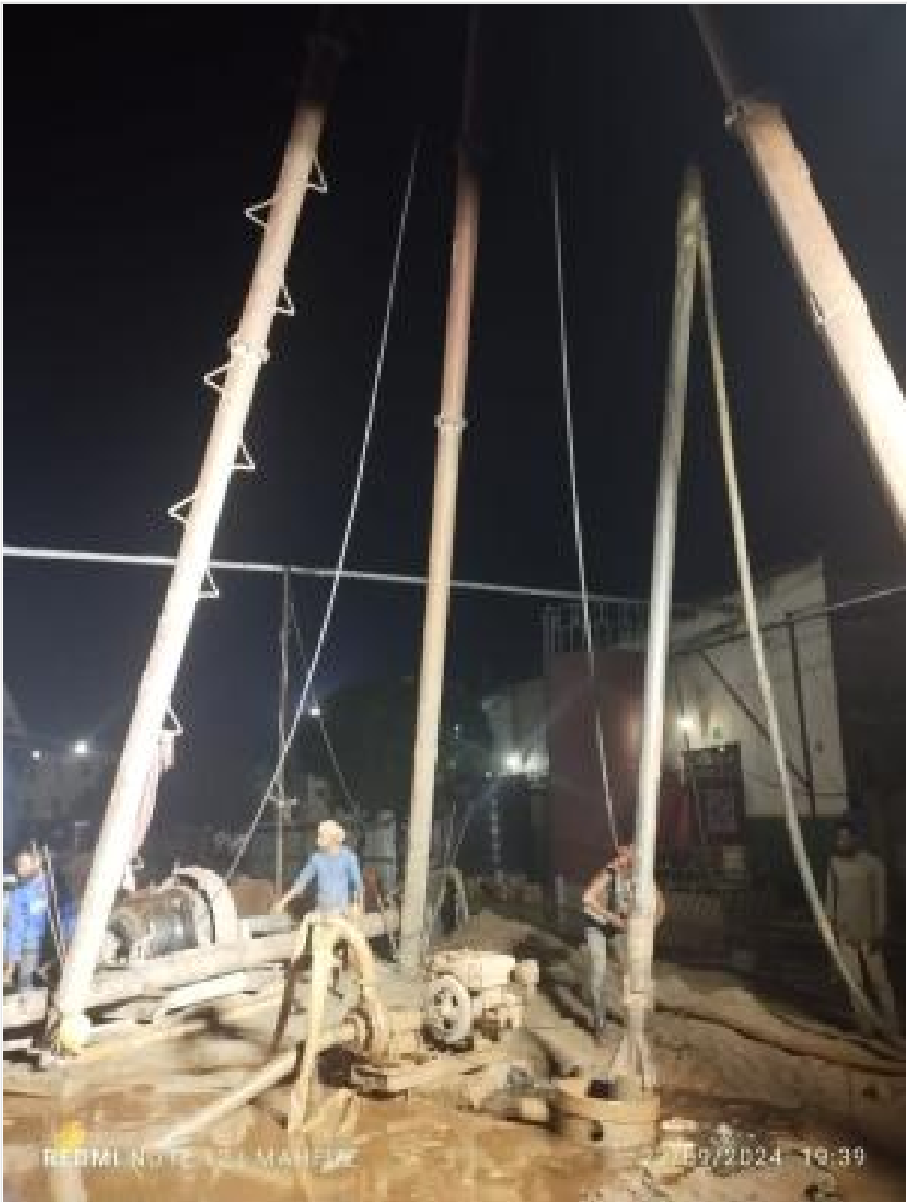
Rig shifting to Grid 1A on 23-09-24
