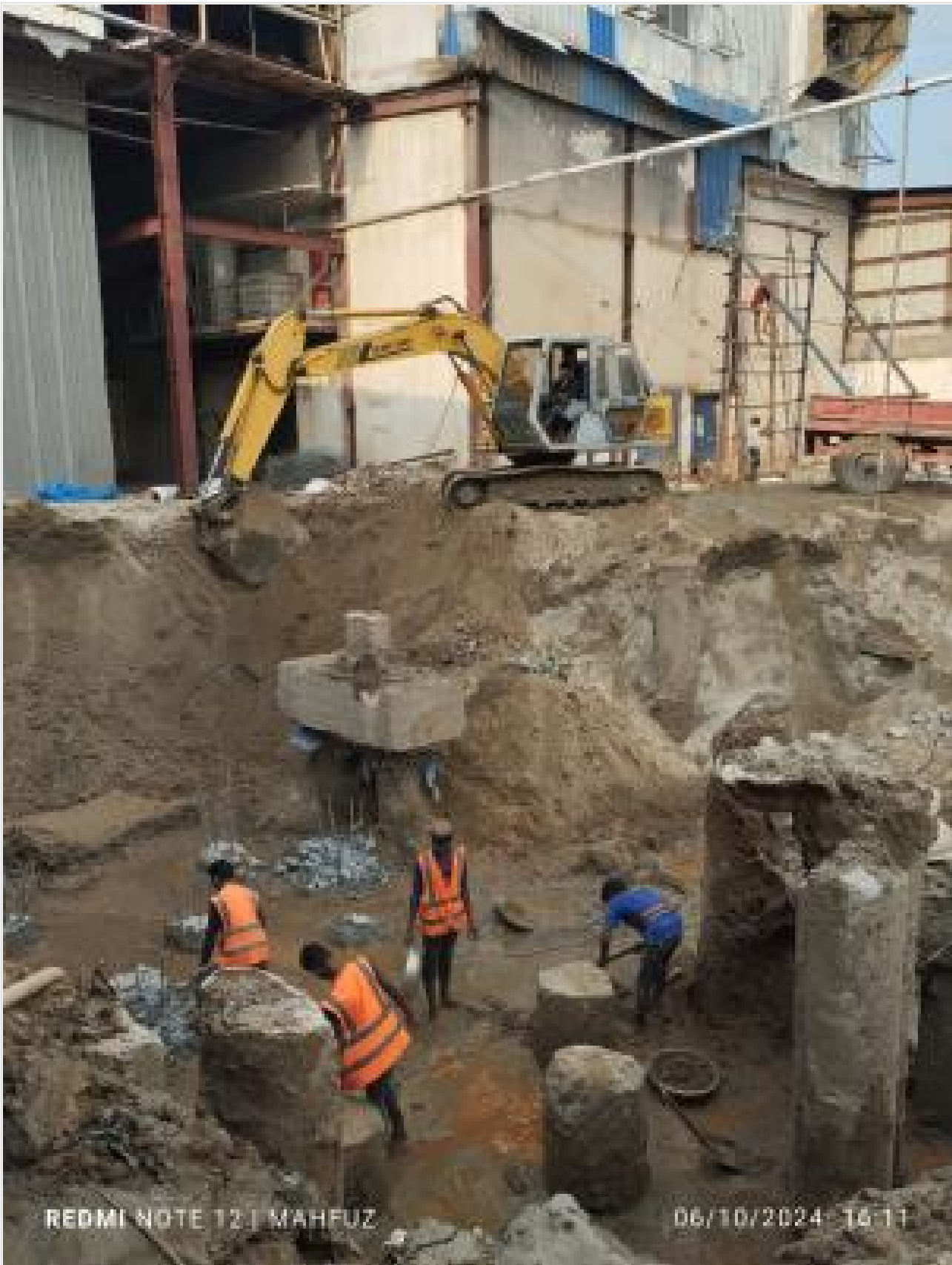
Pile head breaking on 07-10-24
