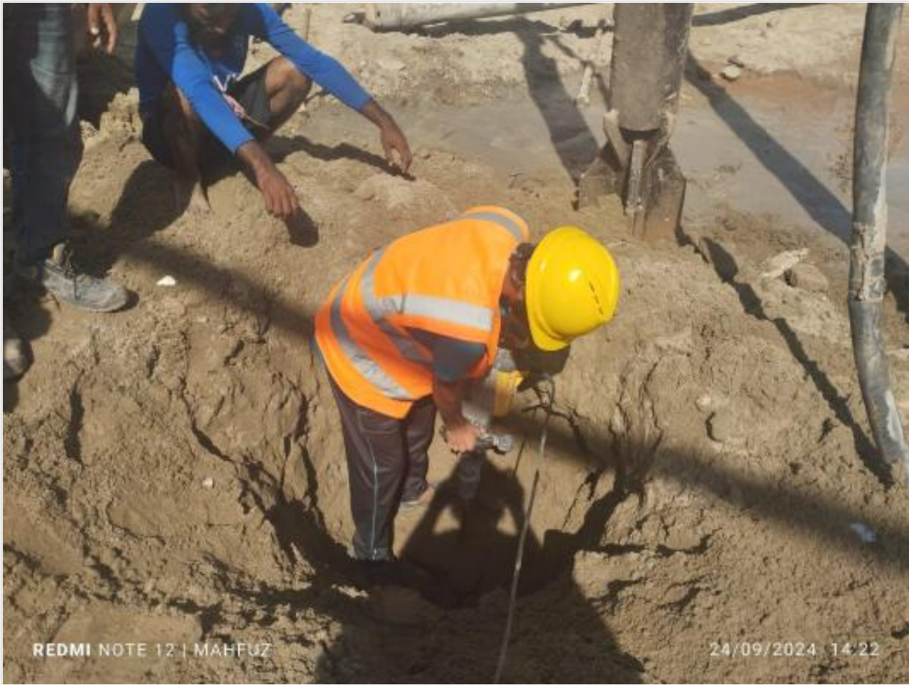
Boring obstacle Old CC breaking on 24-09-24
