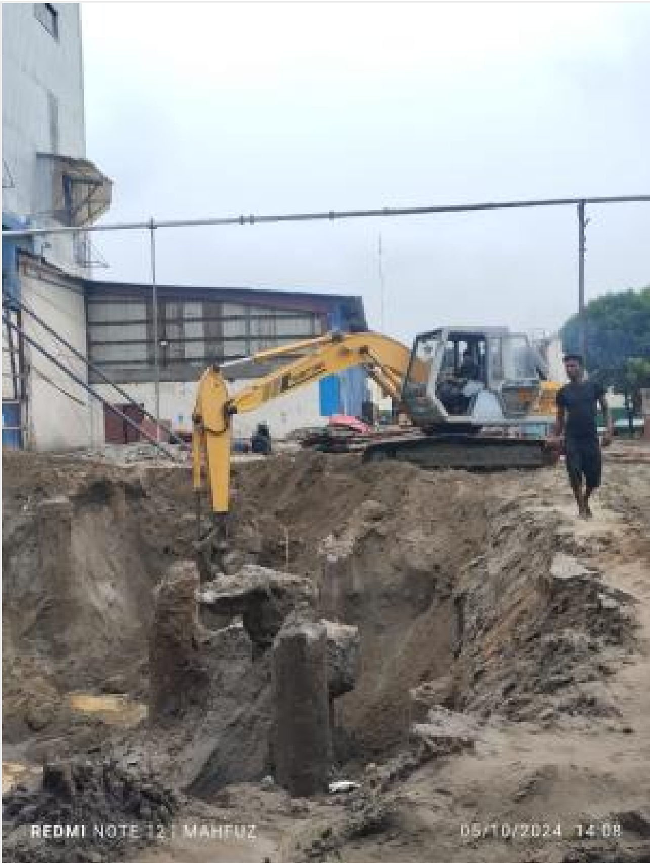
Earth excavation on 05-10-24
