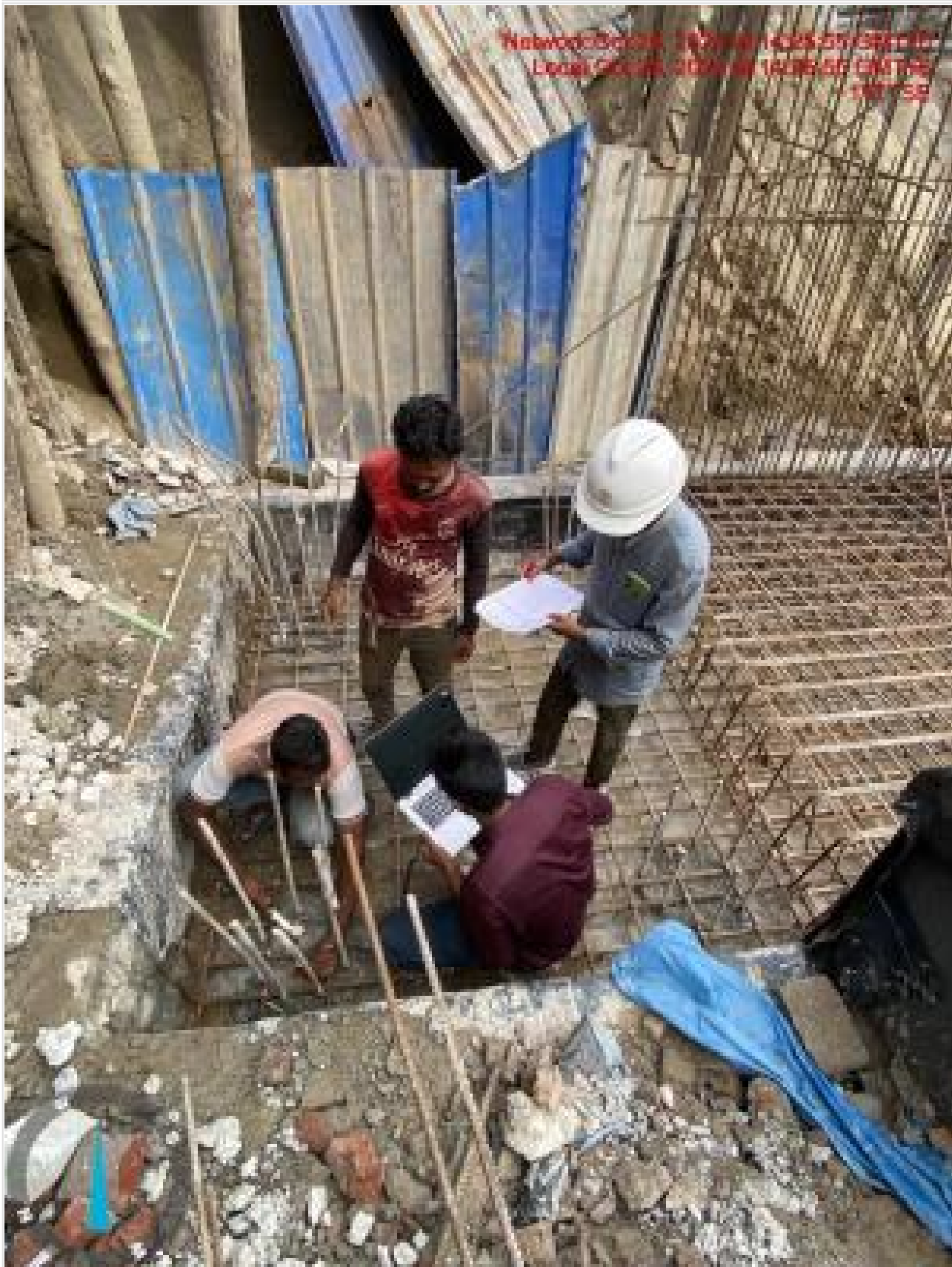
PIT test on 25-10-24
