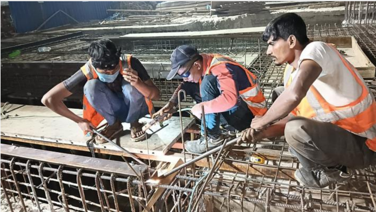
MS Angle Fixing on 24-11-24
