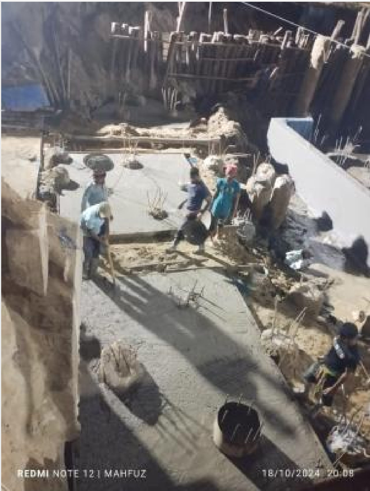
Pile cap lean concreting on 18-10-24
