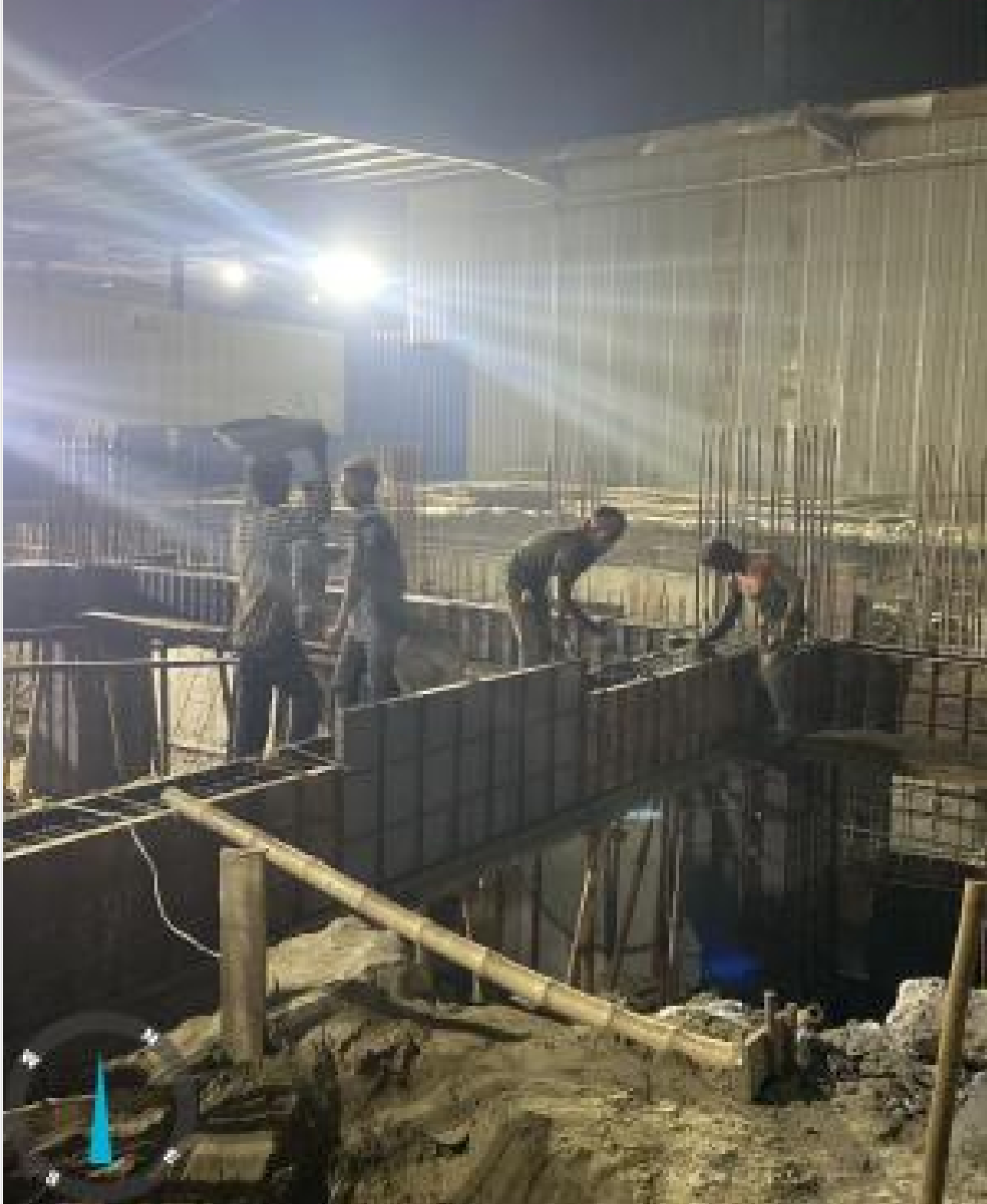
Foundation beam concreting on 12-11-24
