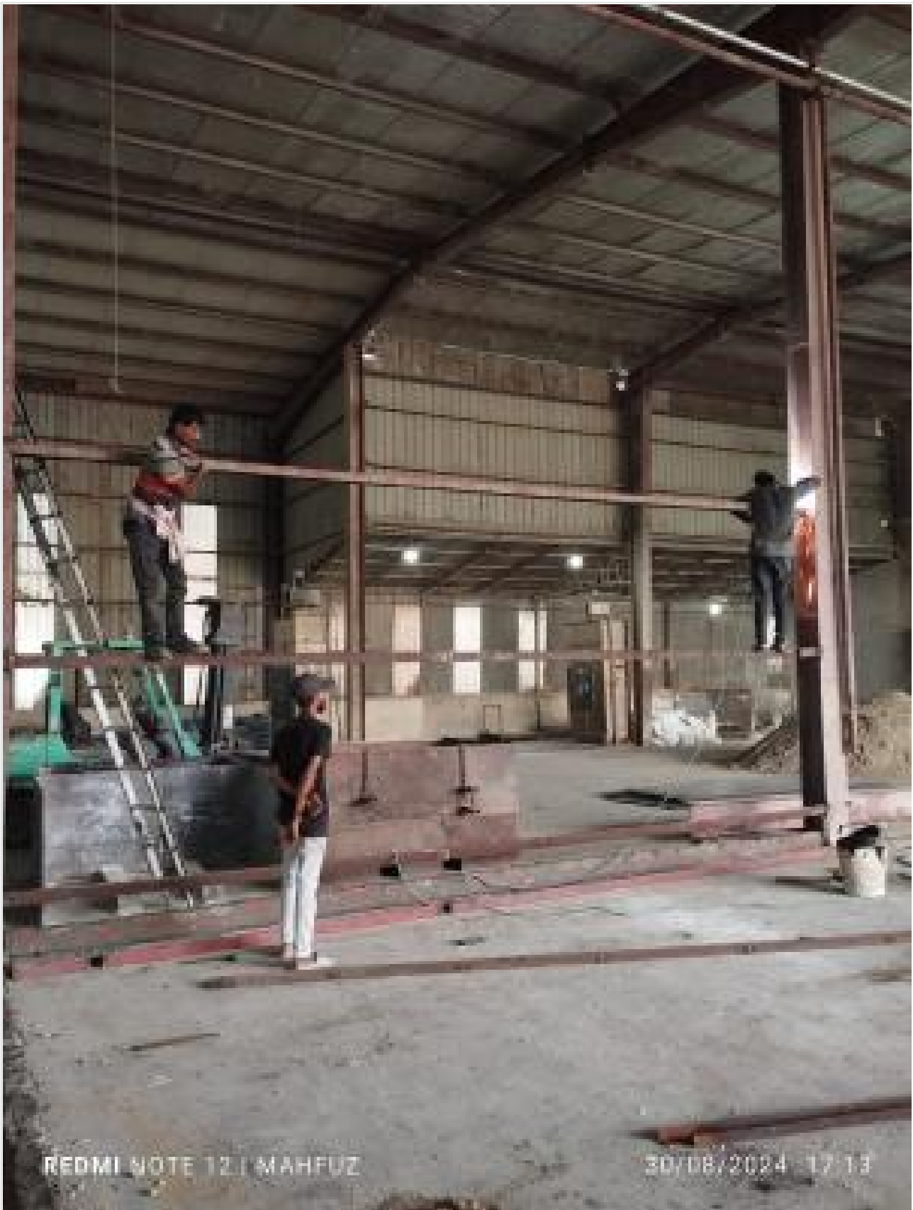
Steel beam cutting on 30-08-24
