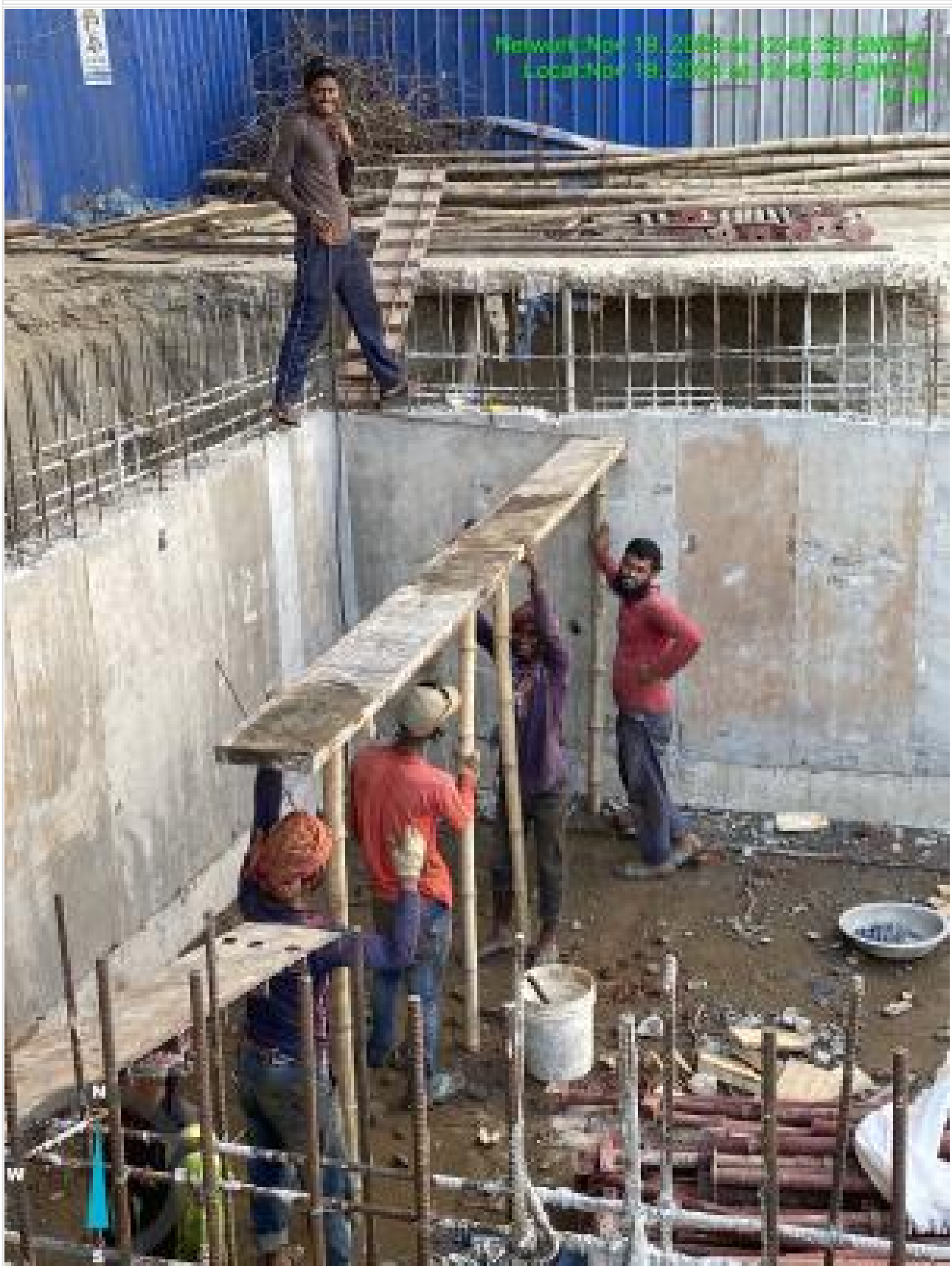
Tank slab shuttering on 19-11-24
