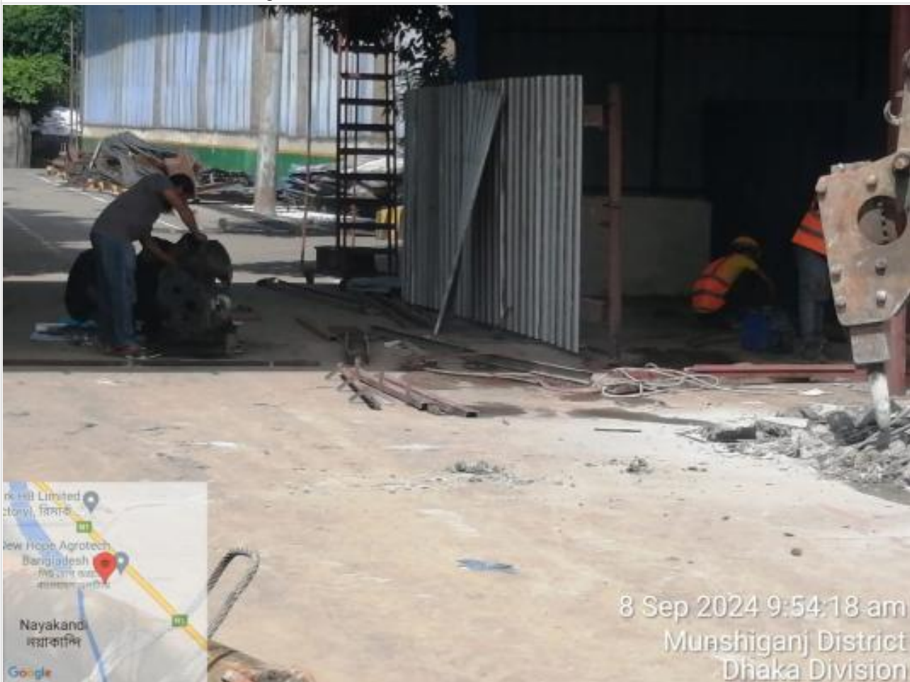
Piling equipment maintenance on 08-09-24
