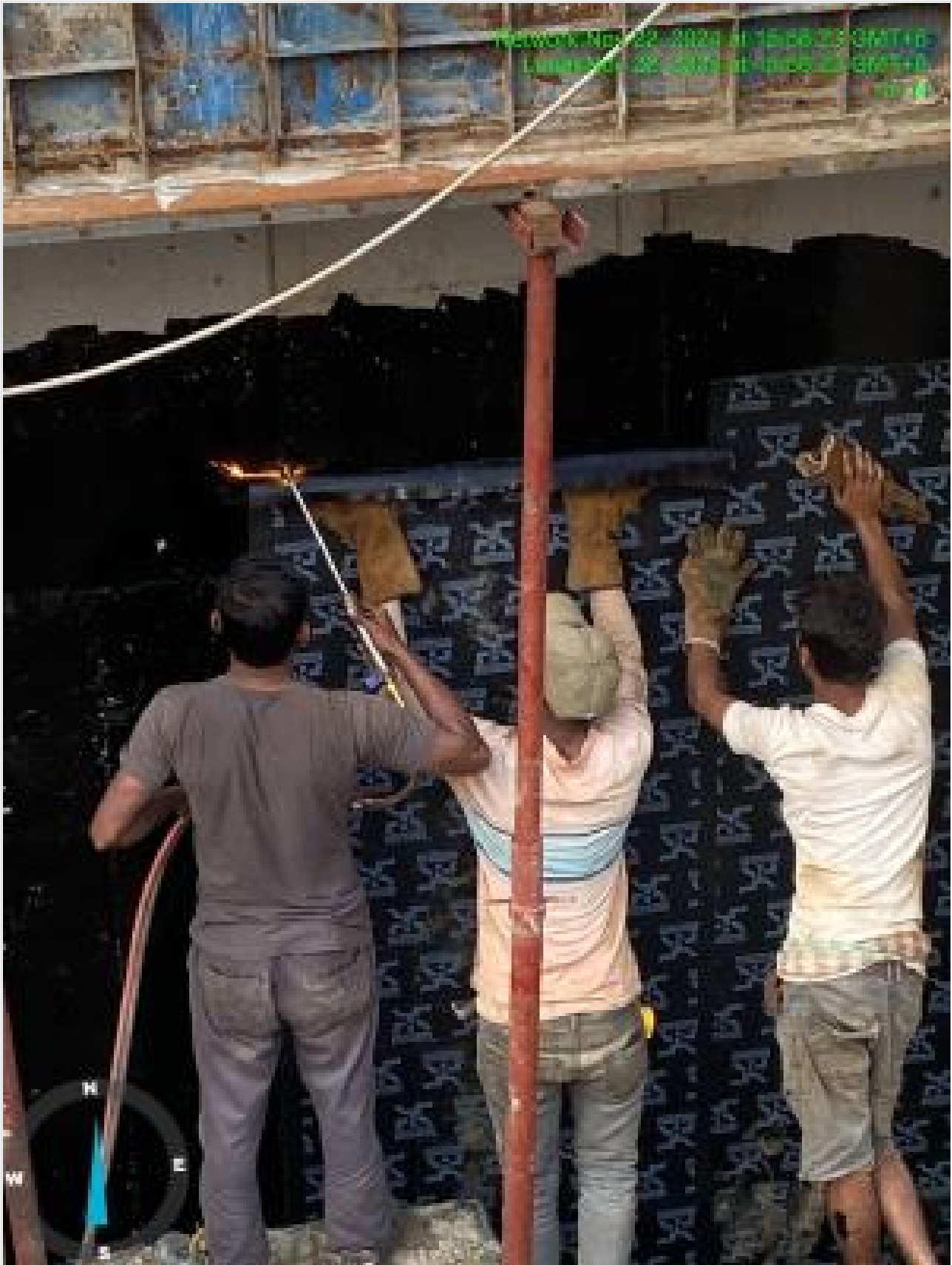
Tank wall water proofing membrain SBS fi on 22-11-24
