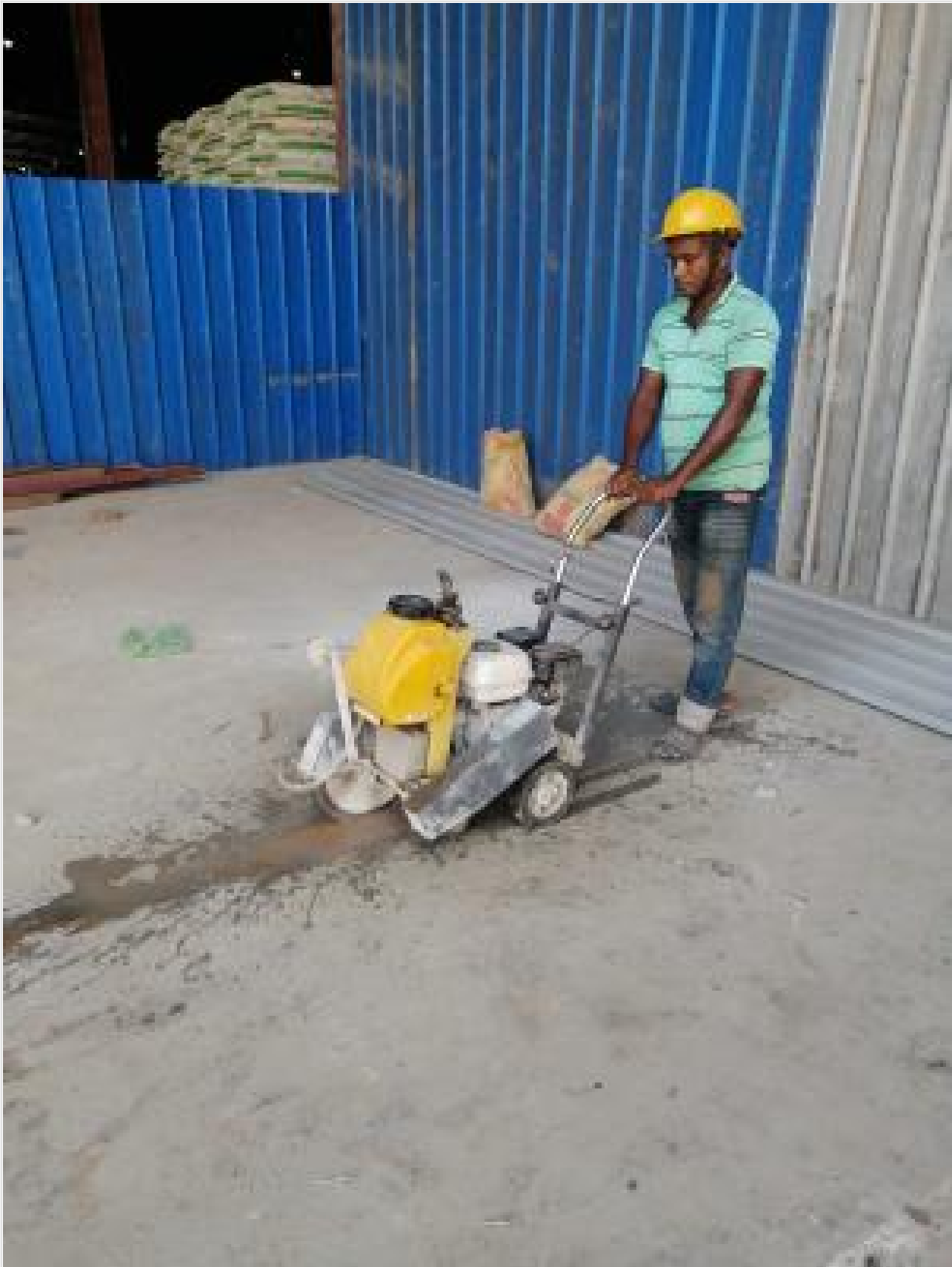
Floor cutting on 02-09-24
