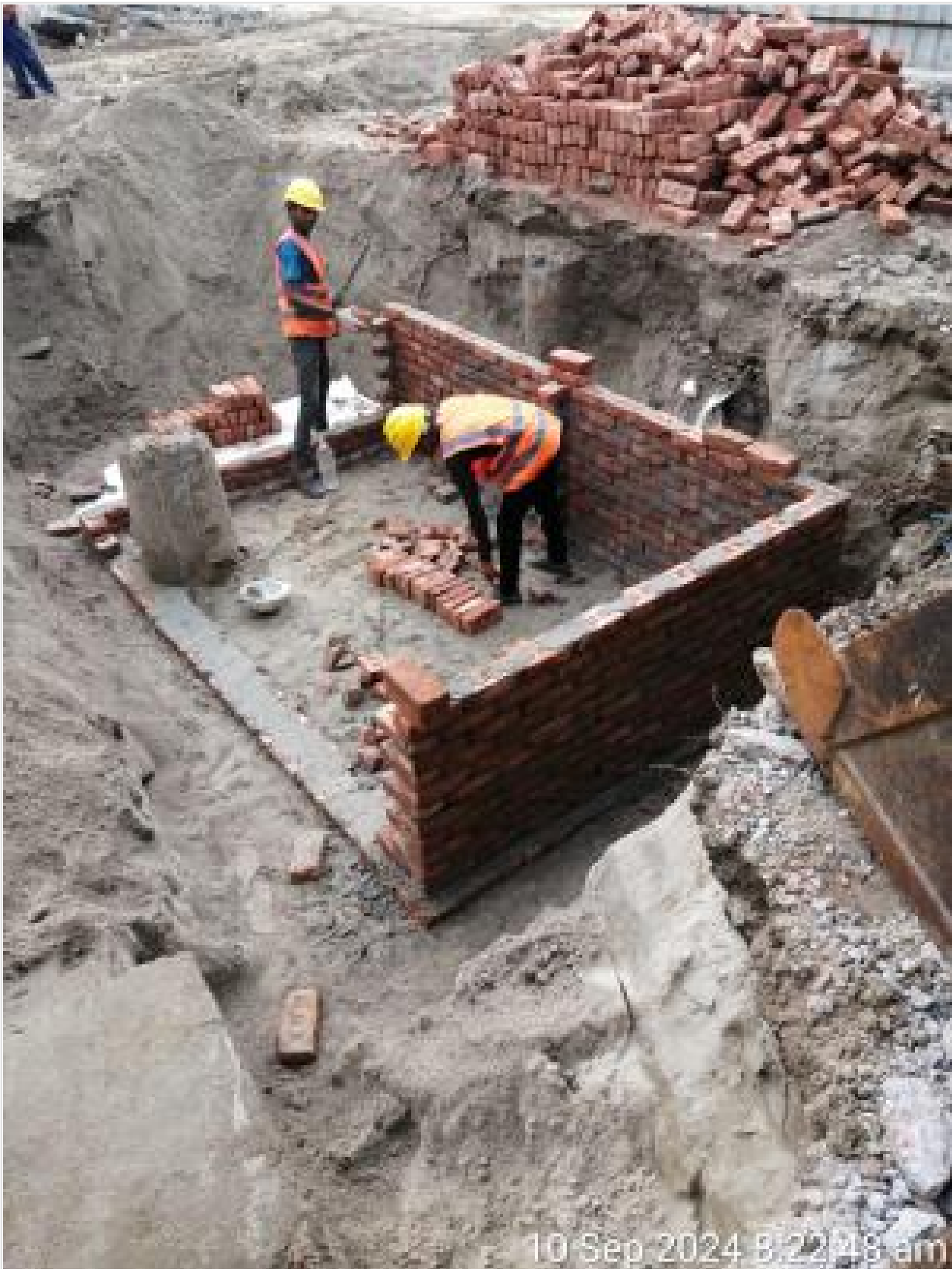
Pile mud tank brick work on 10-09-24
