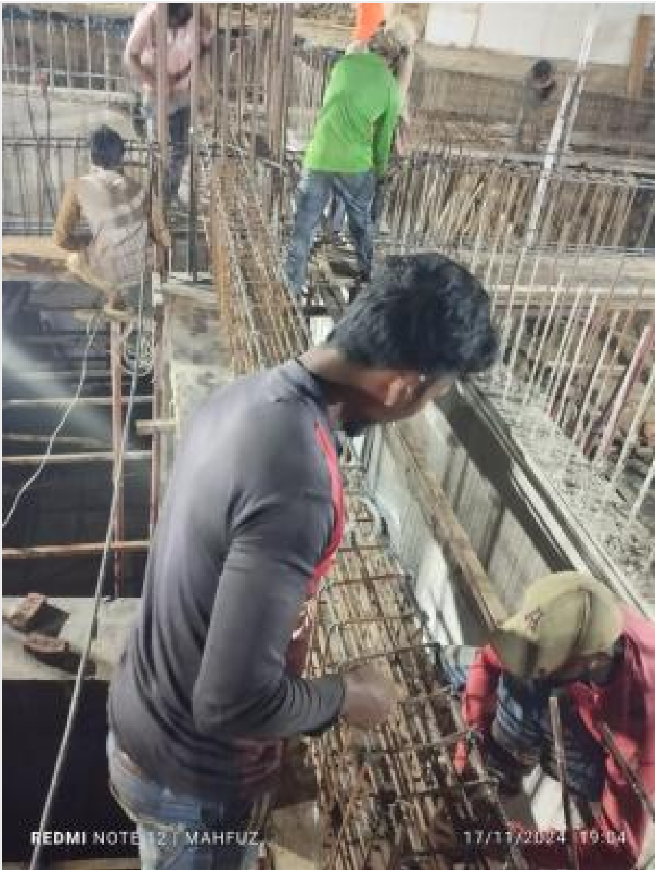
Foundation beam rebar work on 17-11-24
