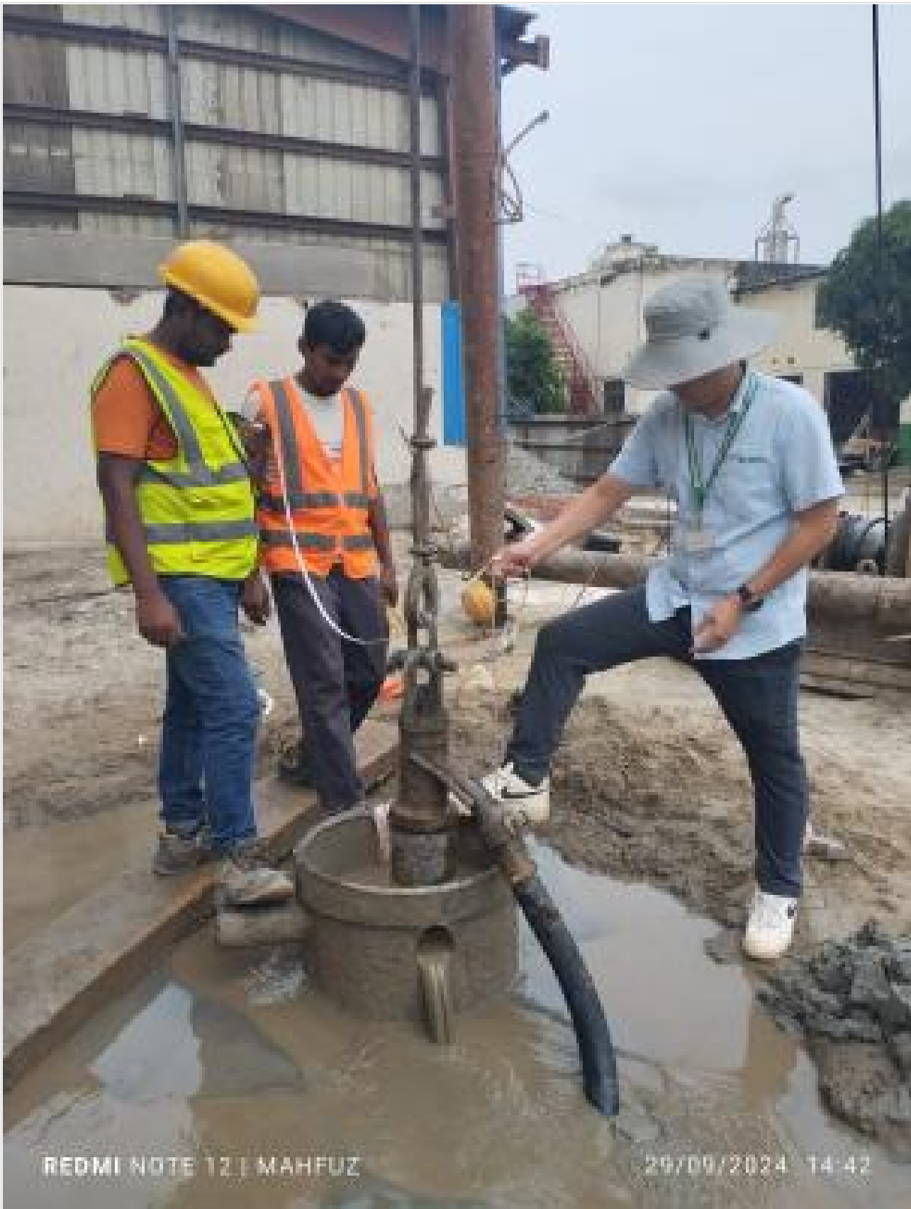
Pile no.47 boring length checking on 29-09-24
