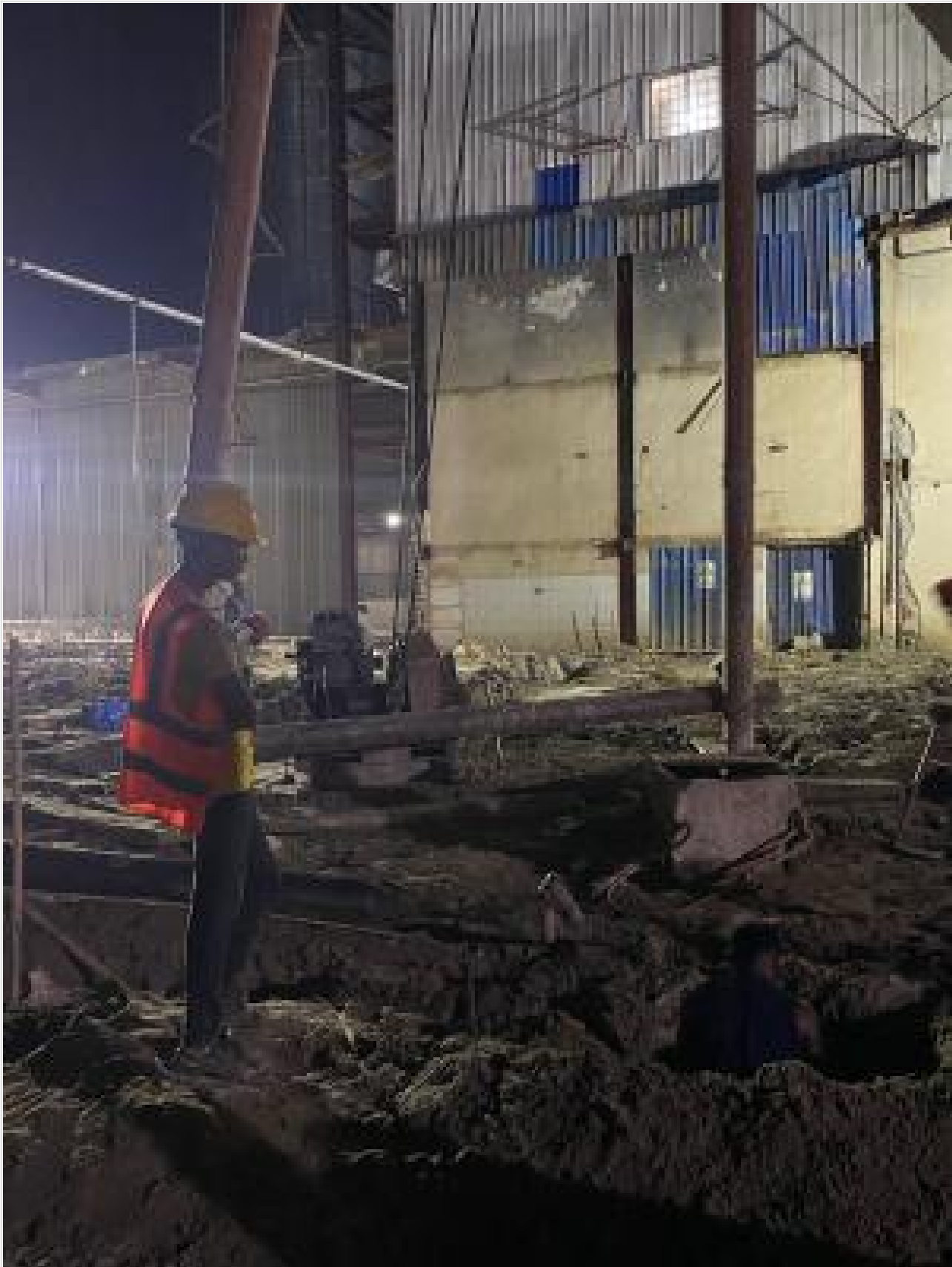
Piling rig shifting on 28-09-24
