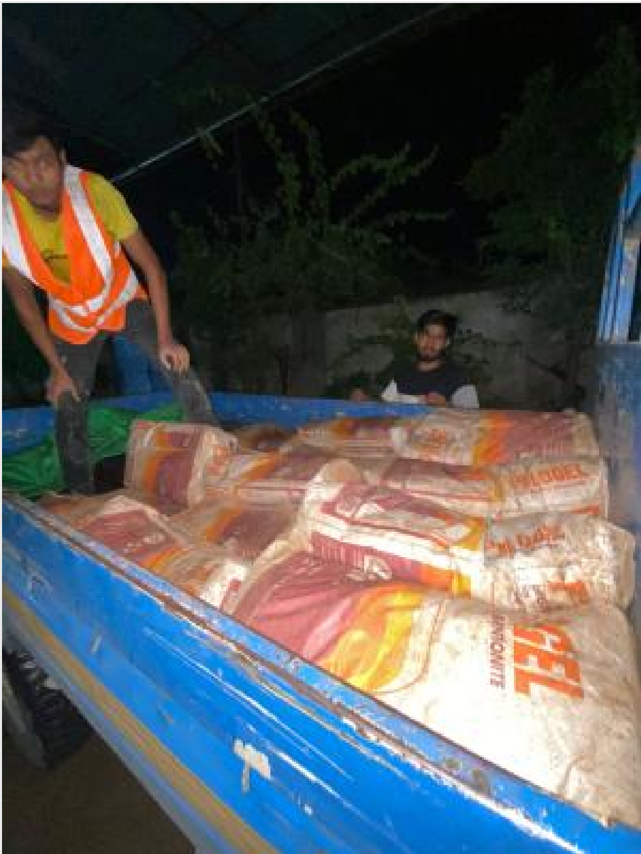
Bentonite received for pile boring on 26-09-24
