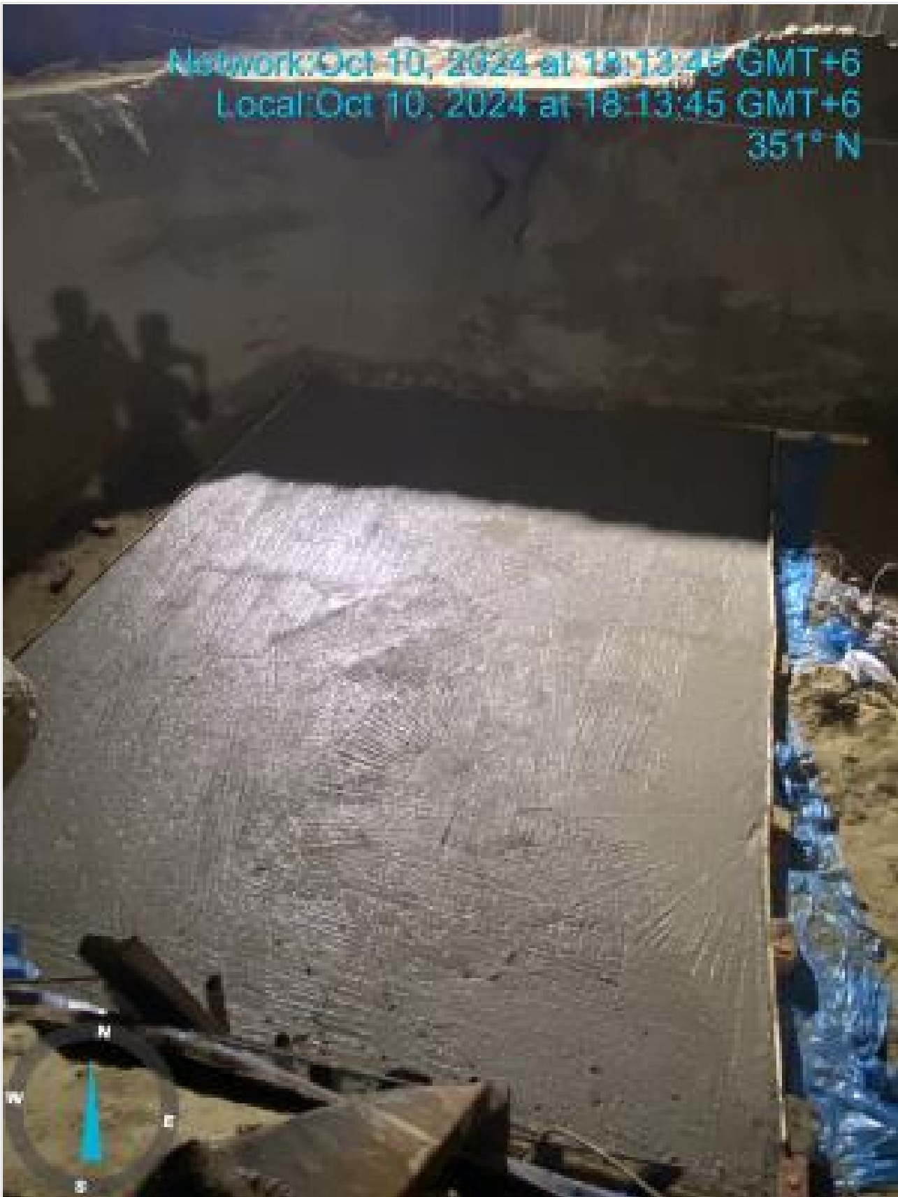
Water Reservoir Base CC-Bottom on 10-10-24
