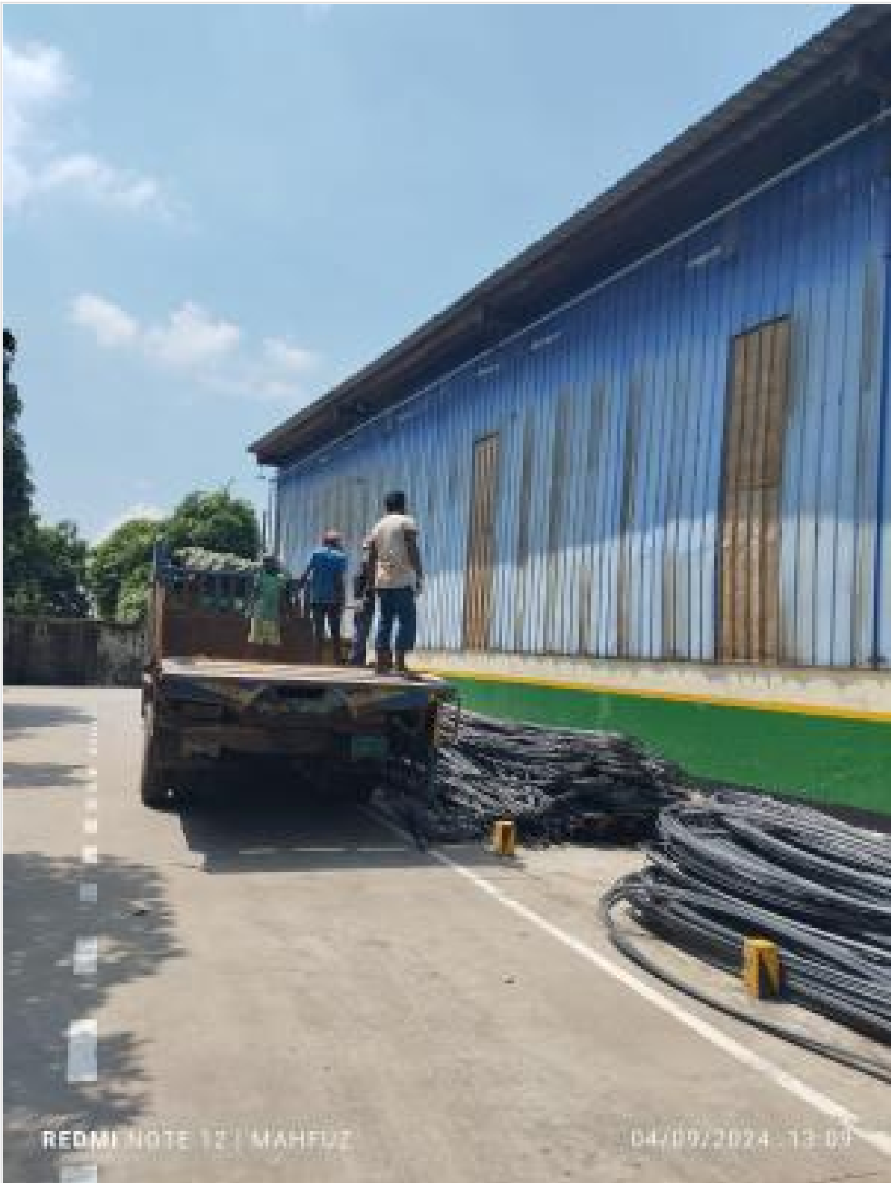
Pile Re-bar mobilized on 04-09-24
