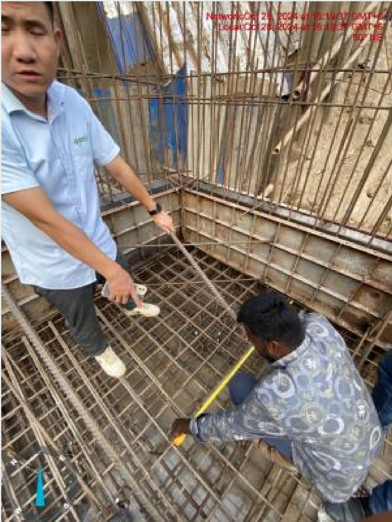
Raft re-bar inspection before concreting on 28-10-24
