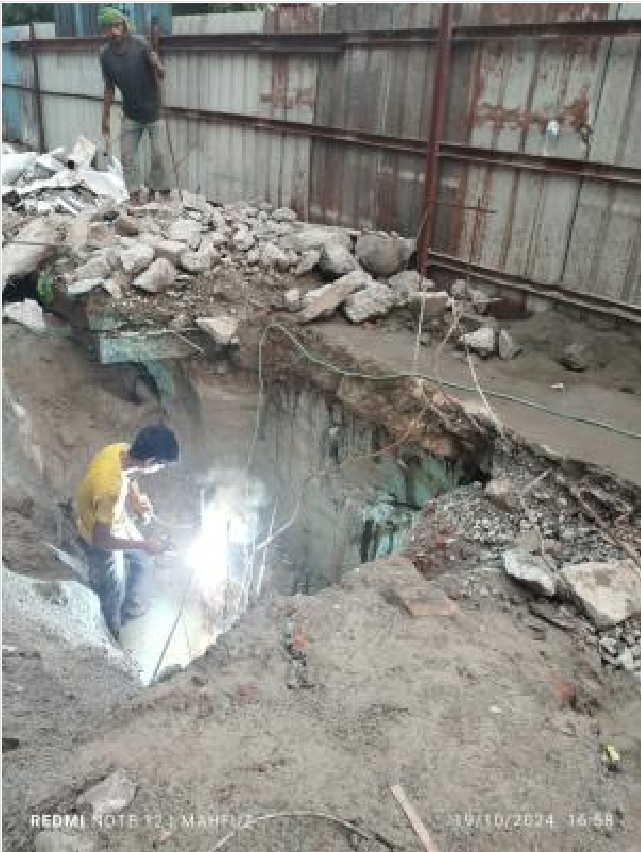
Pile Head Breaking on 19-10-24
