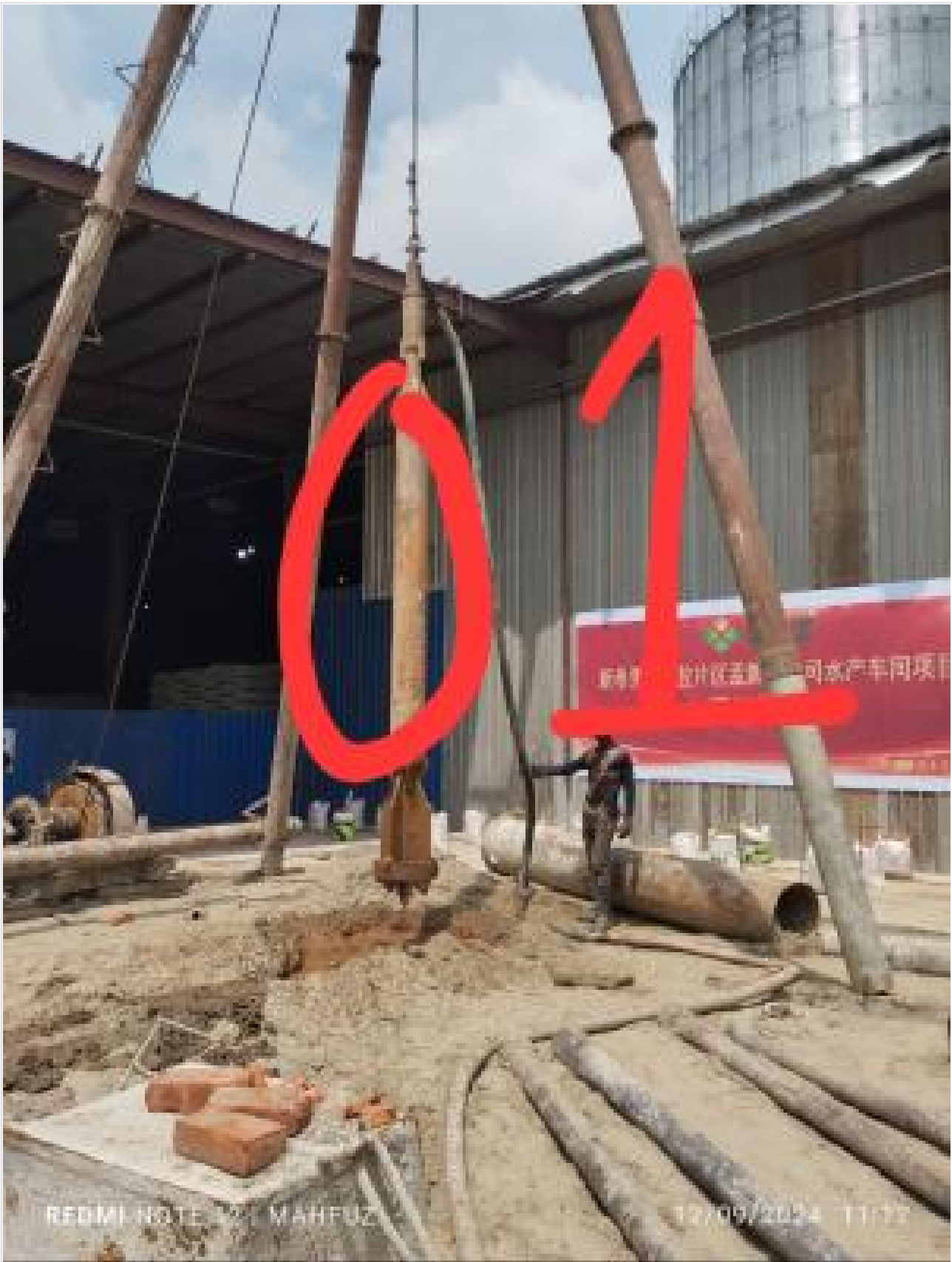
Pile boring on 12-09-24
