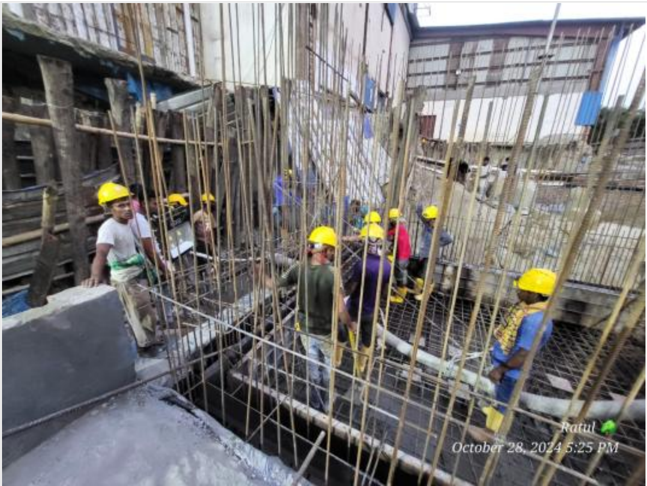
Raft concreting by Pump on 28-10-24
