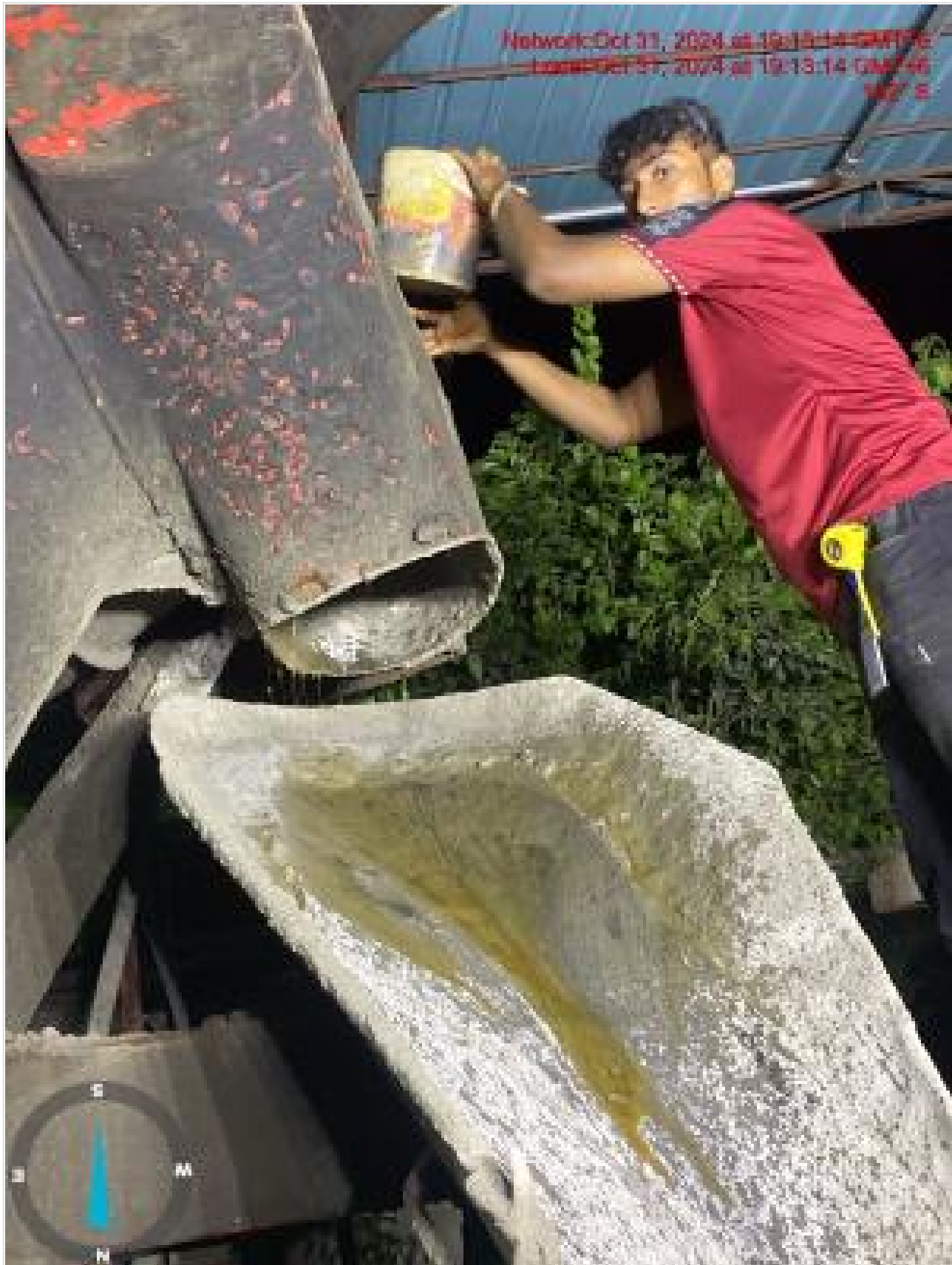
Water proofing admixture adding in concr on 31-10-24
