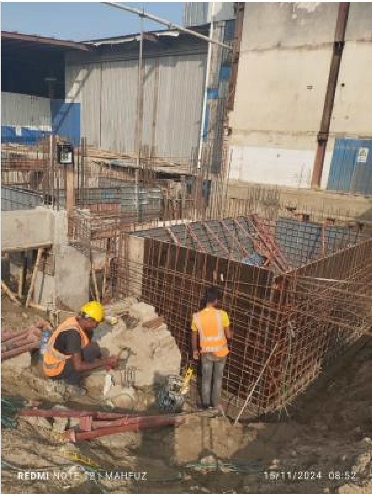
Wall shuttering on 15-11-24
