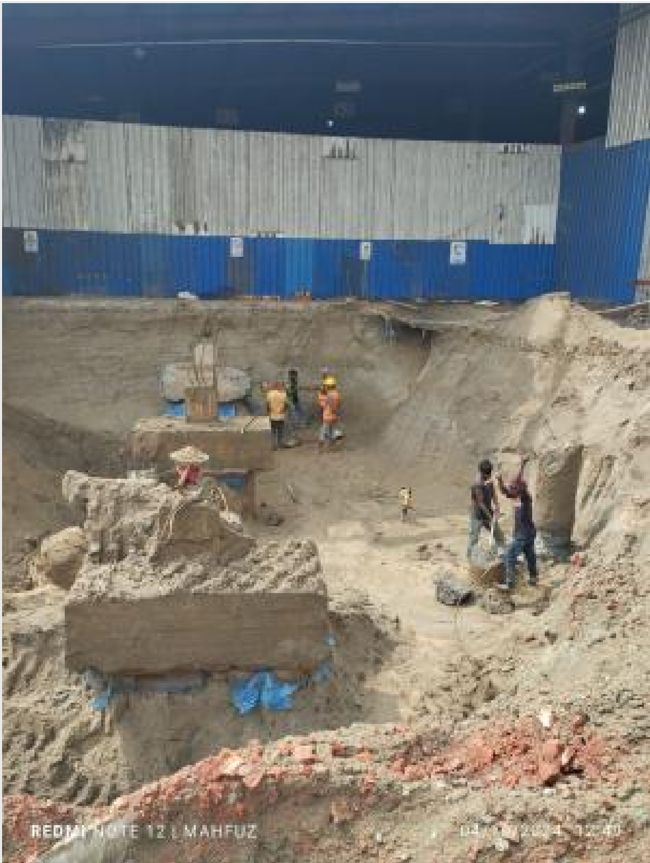
Pile Head breaking on 04-10-24
