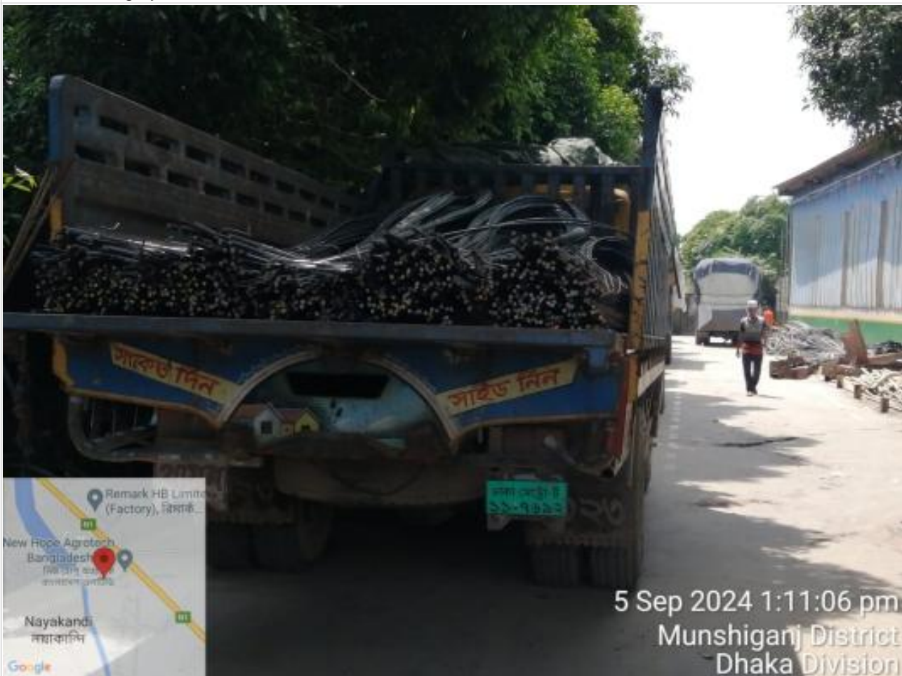
Pile re-bar mobilized on 05-09-24
