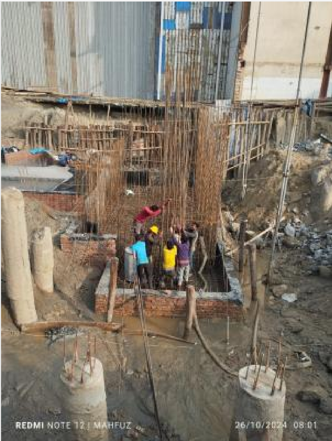
Column re-bar work on 26-10-24
