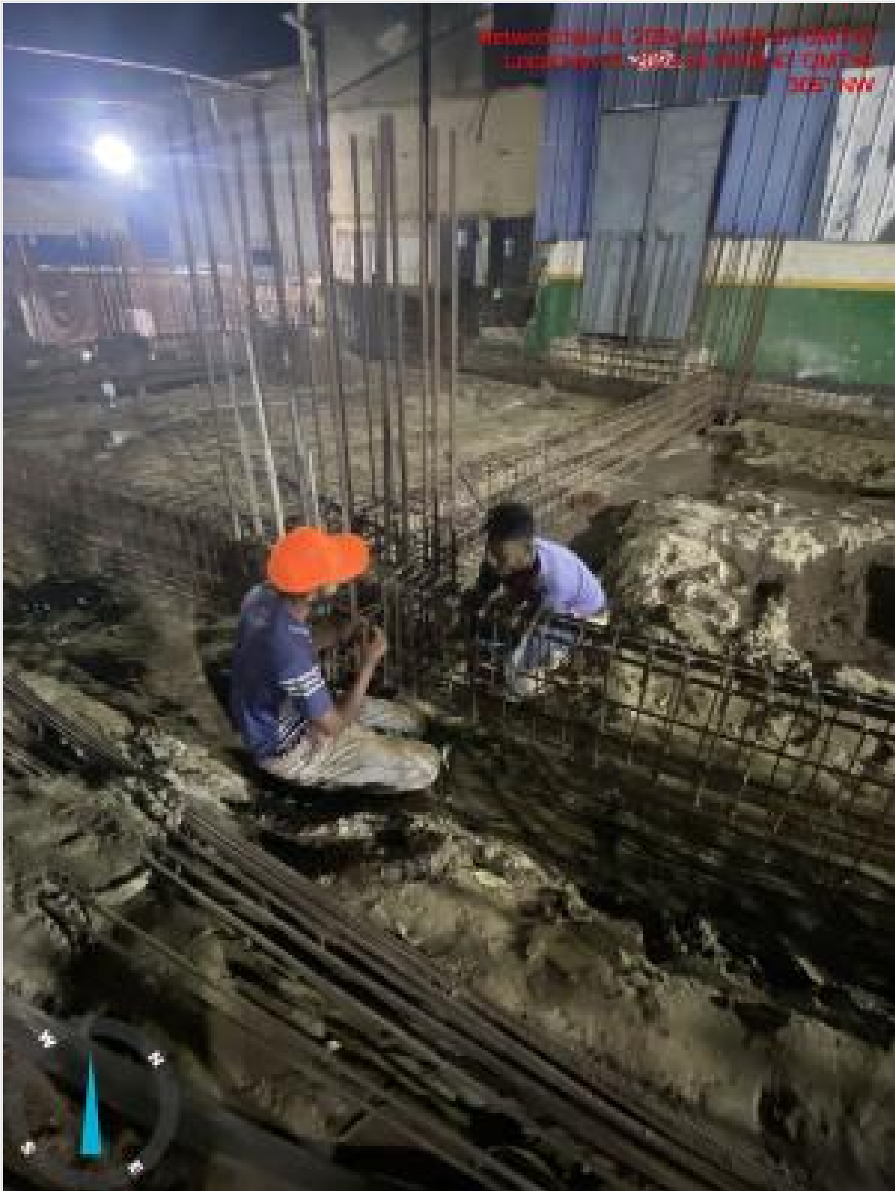
Foundation beam rebar work on 08-11-24
