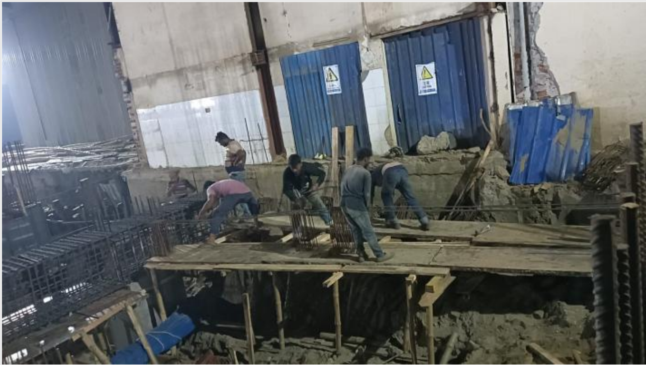
Foundation beam rebar work on 15-11-24
