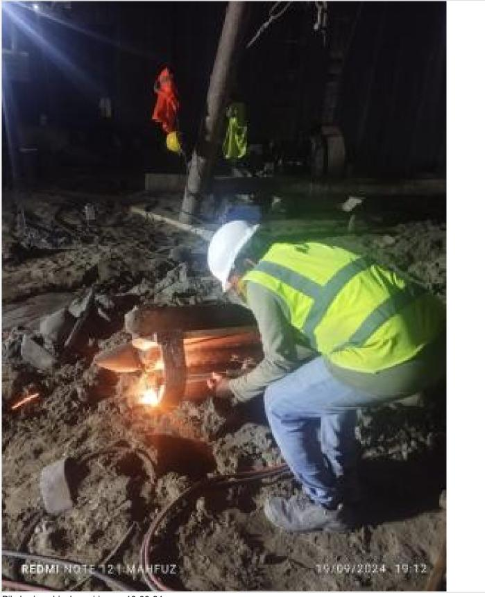
Pile boring chisel repairing on 19-09-24
