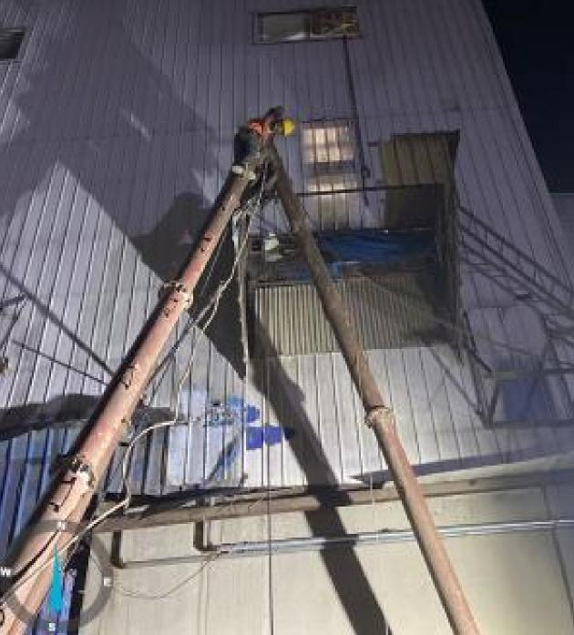
Piling rig setting on 29-09-24 Pile no.47 of grid 3C length 22m Total 6 piles 22 m
