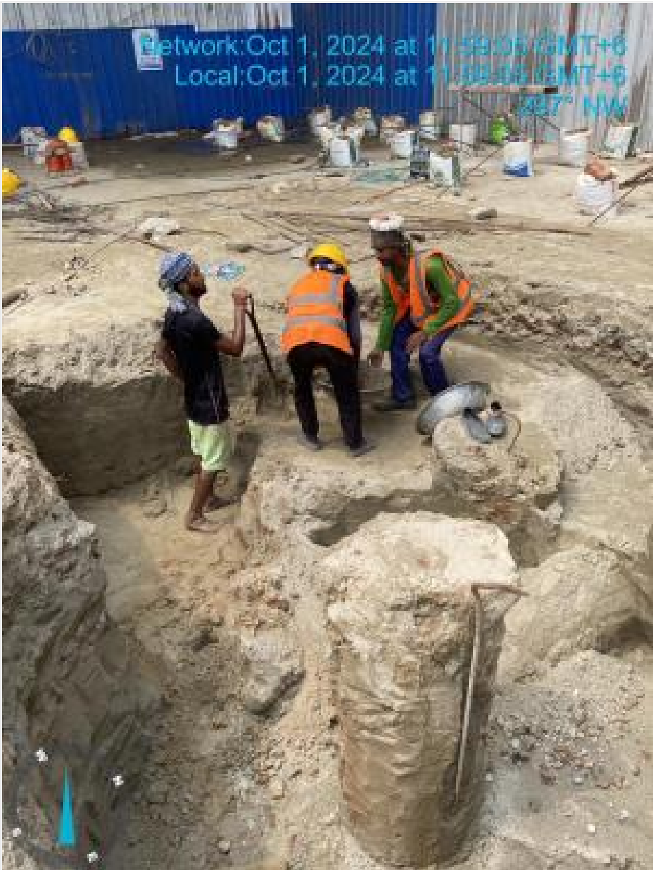
Earth excavation on 01-10-24
