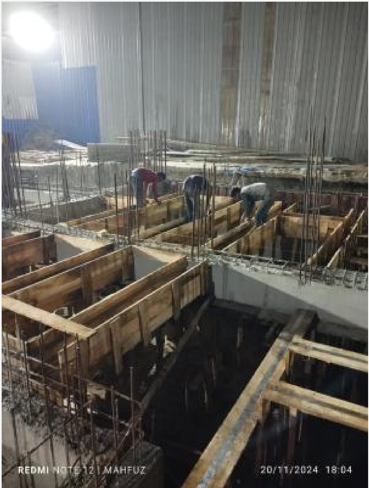
Tank slab shuttering on 20-11-24
