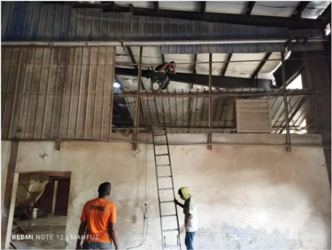
Sheet removing on 28-08-24
