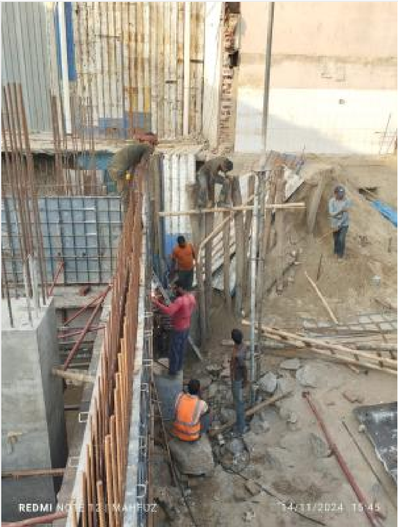
Wall shuttering on 14-11-24
