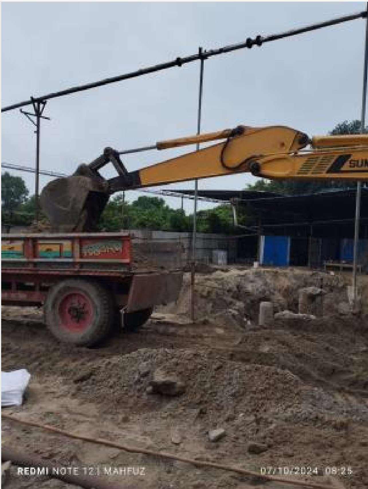
Earth excavation on 07-10-24
