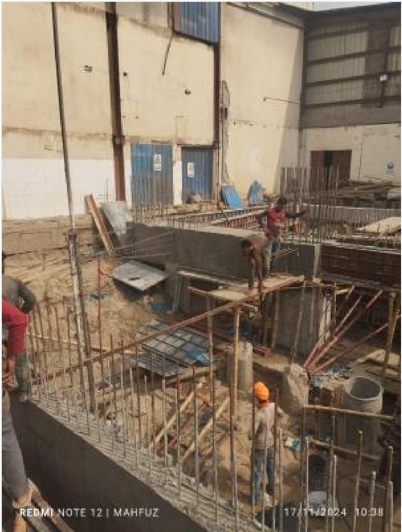
Foundation beam bottom shuttering on 17-11-24
