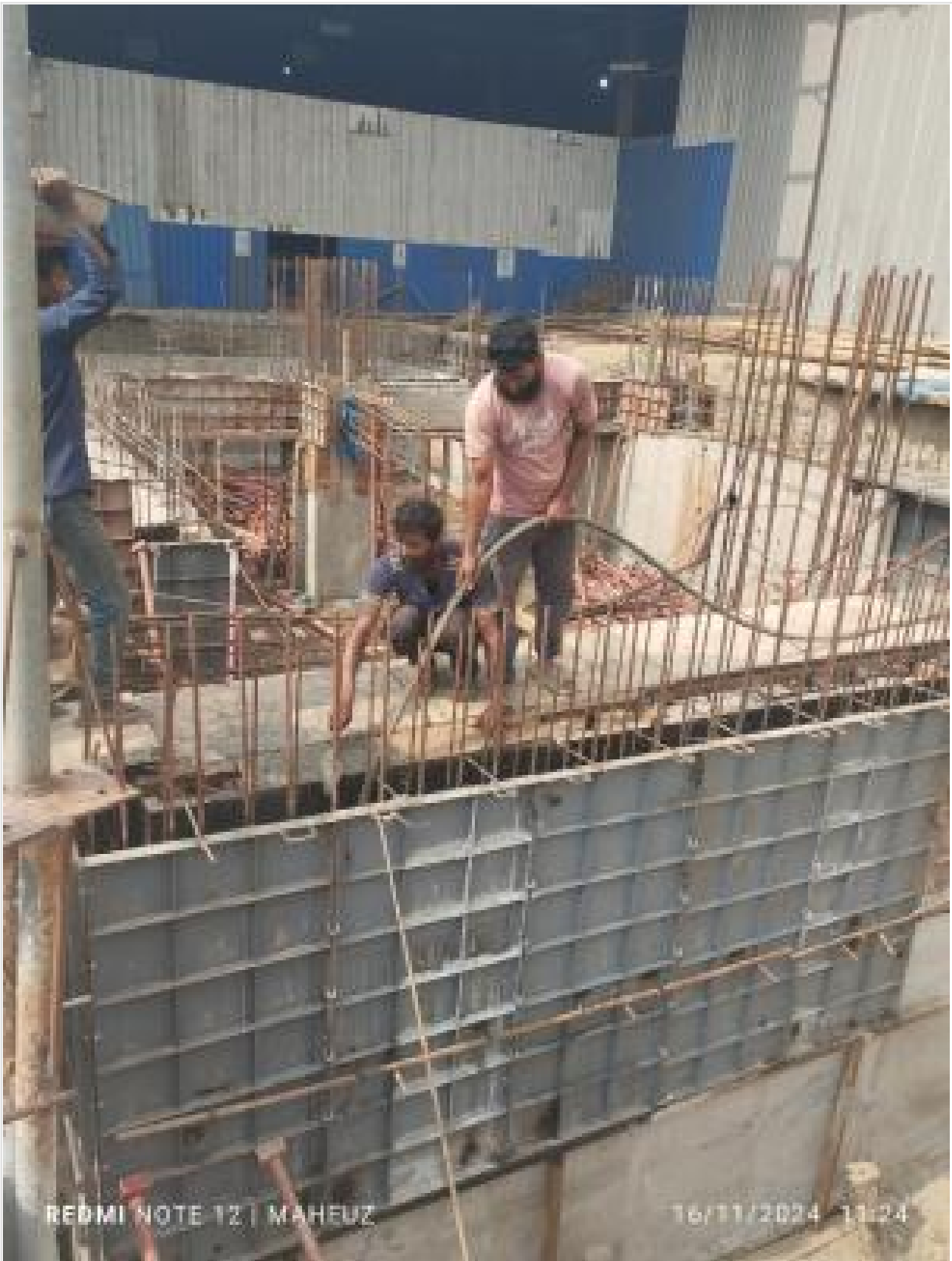
Wall concreting on 16-11-24
