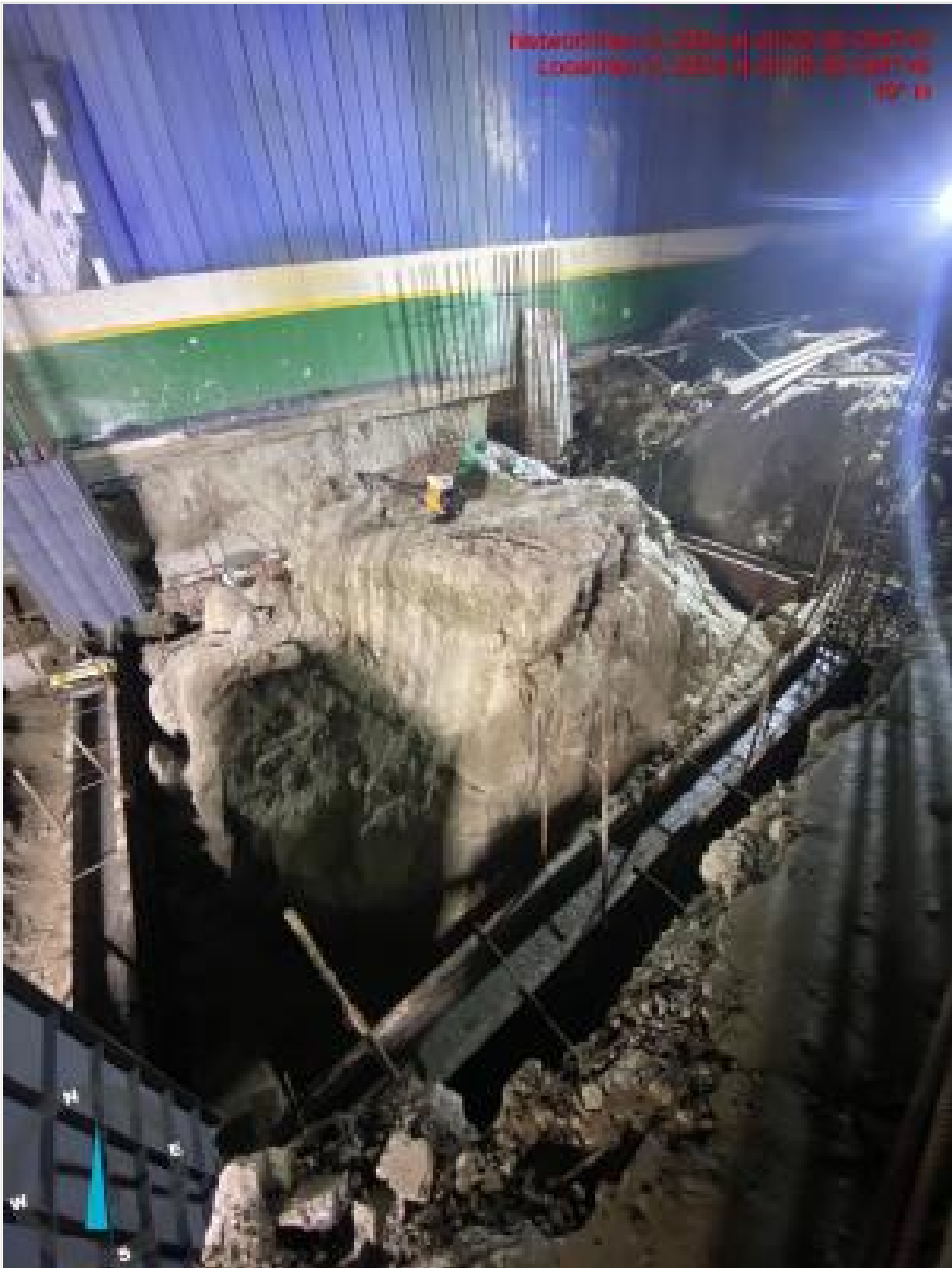
Bracing beam concreting on 02-11-24
