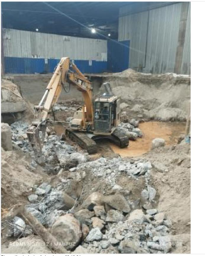
Dismantling by hydraulic breaker on 08-10-24 Dismantling old foundation 17 m3 By Hydraulic hammer
