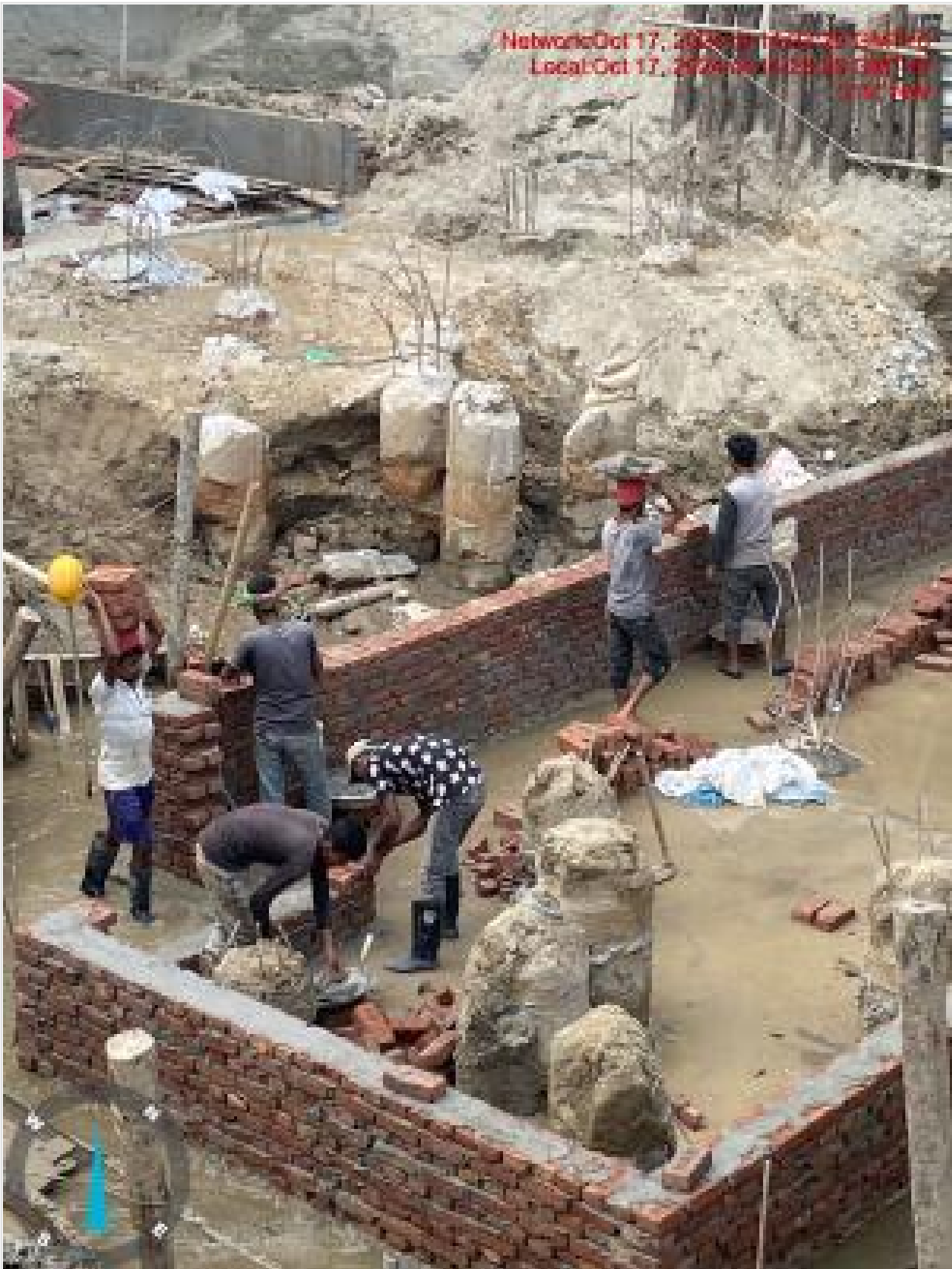
Water tank base brick wall shuttering on 17-10-24
