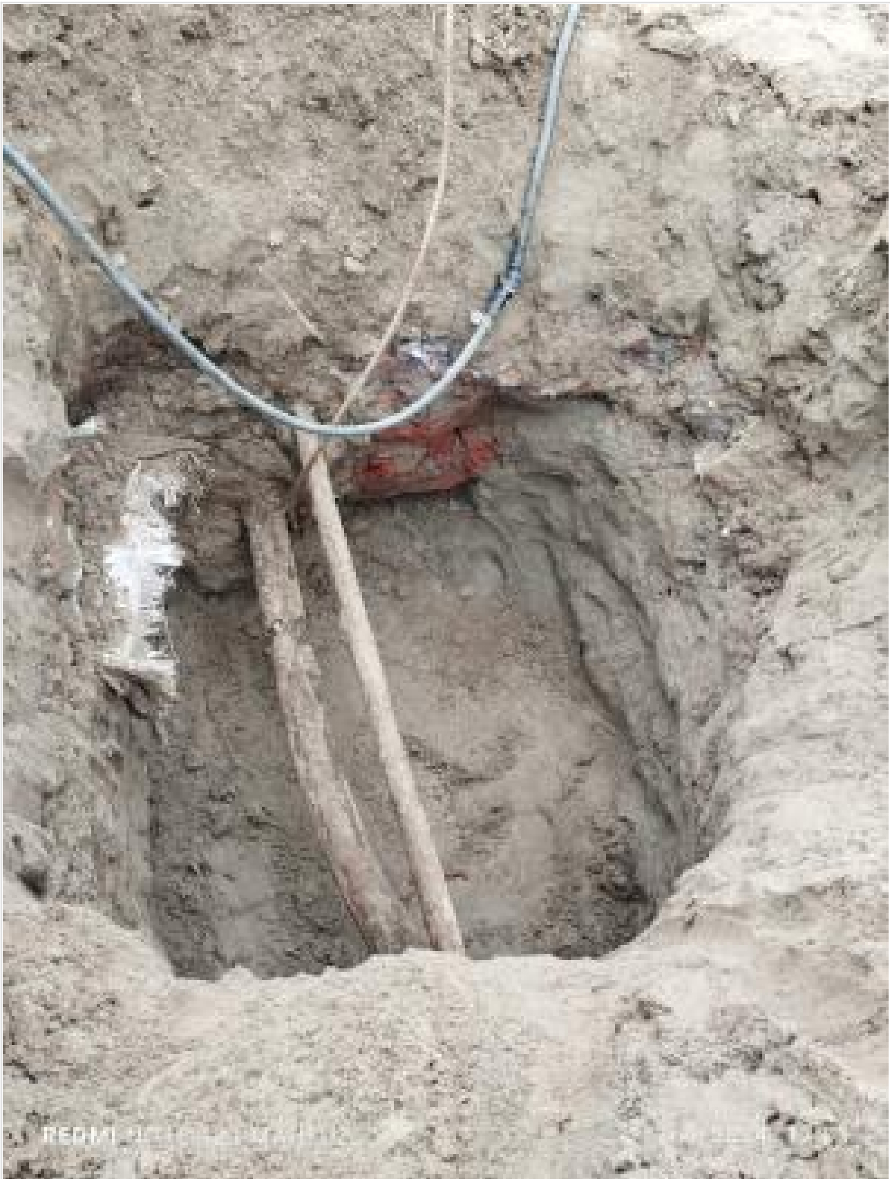
During boring Obstacles found on 21-09-24
