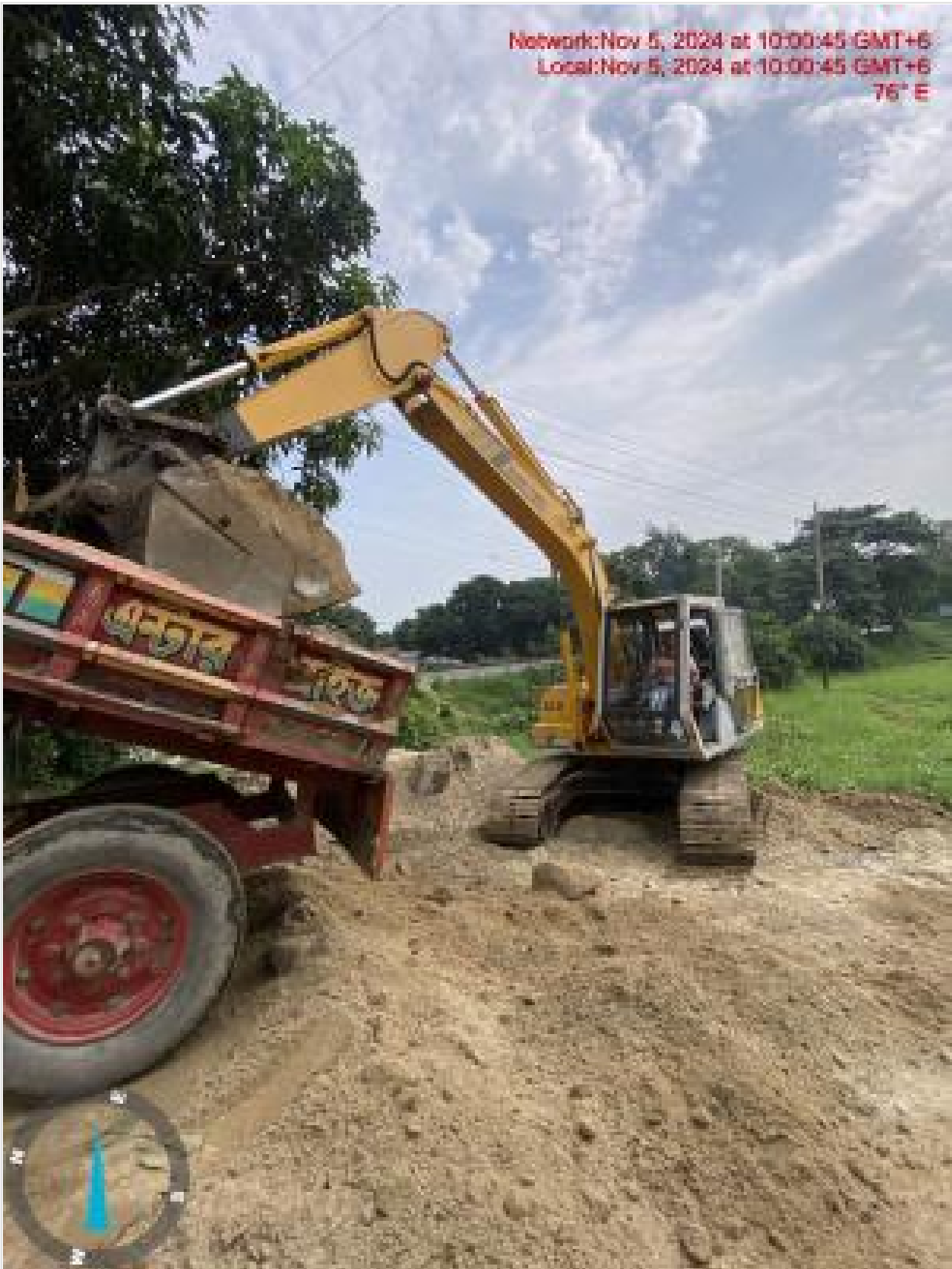
Earth loading for backfilling on 05-11-24
