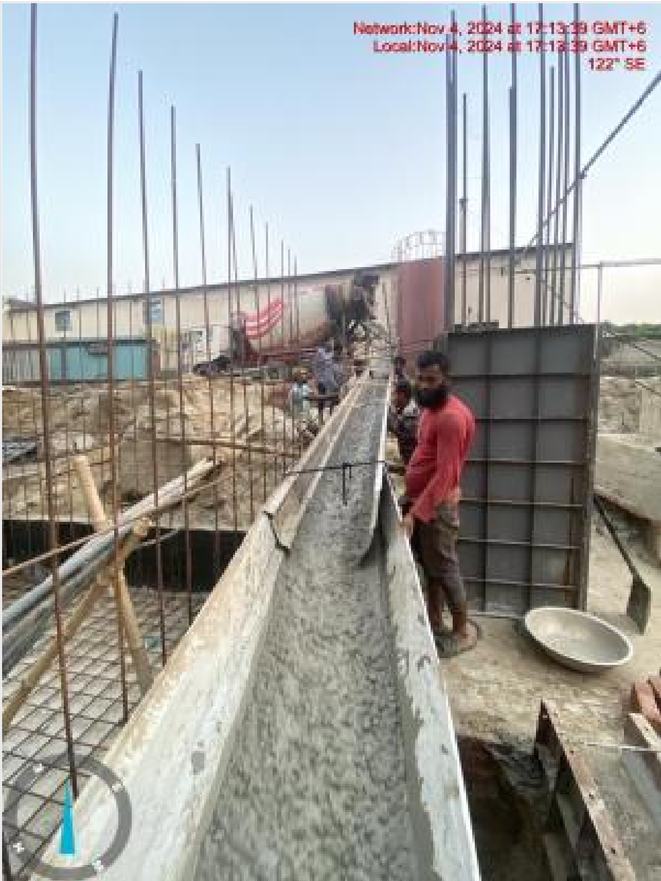
Pile cap Concreting on 04-11-24
