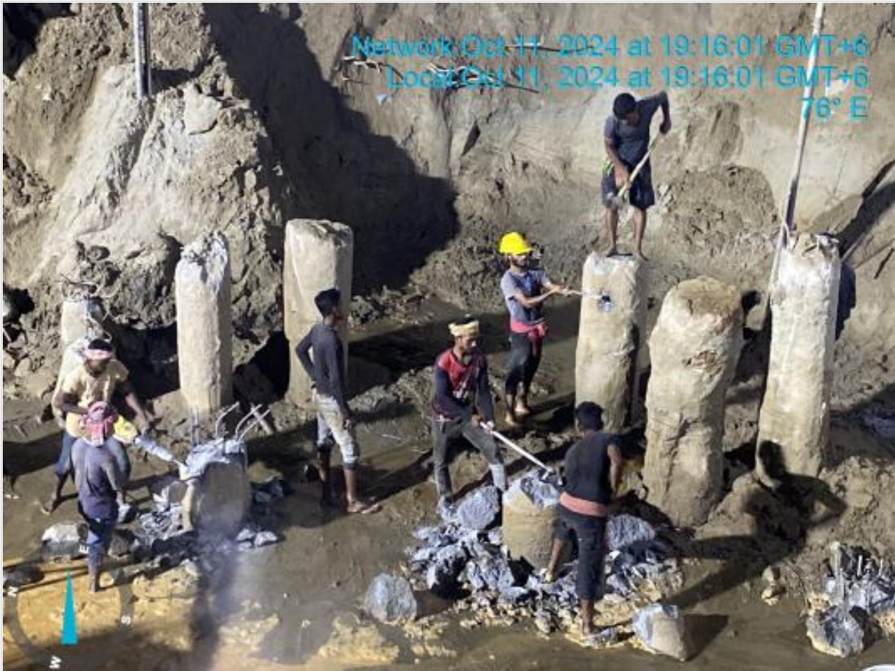
Pile head breaking on 11-10-24
