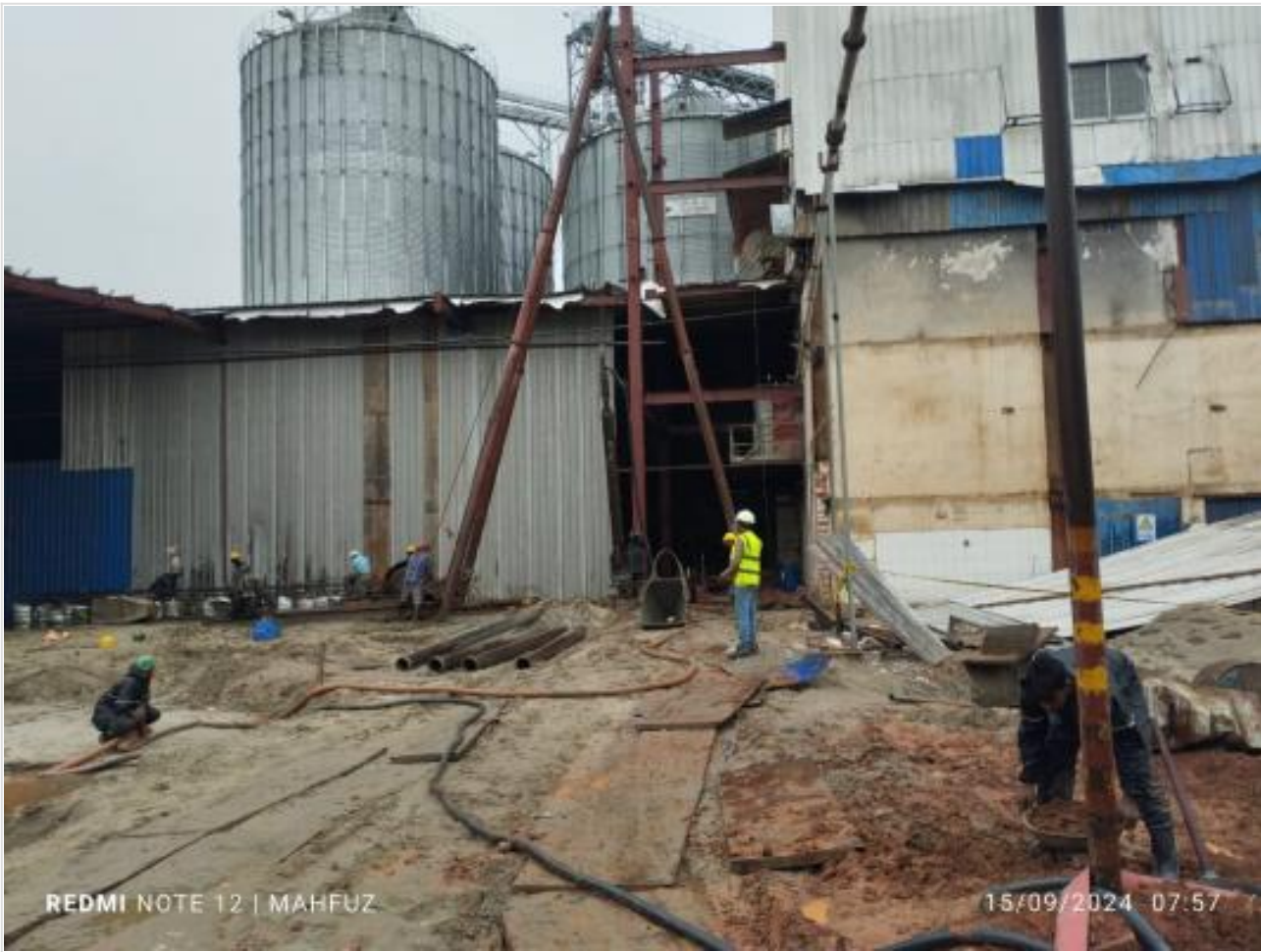
Pile boring on 15-09-24
