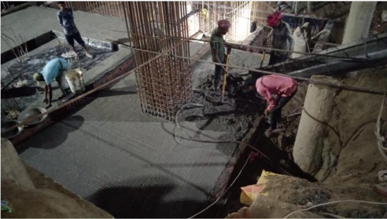
Pile cap concreting on 25-10-24
