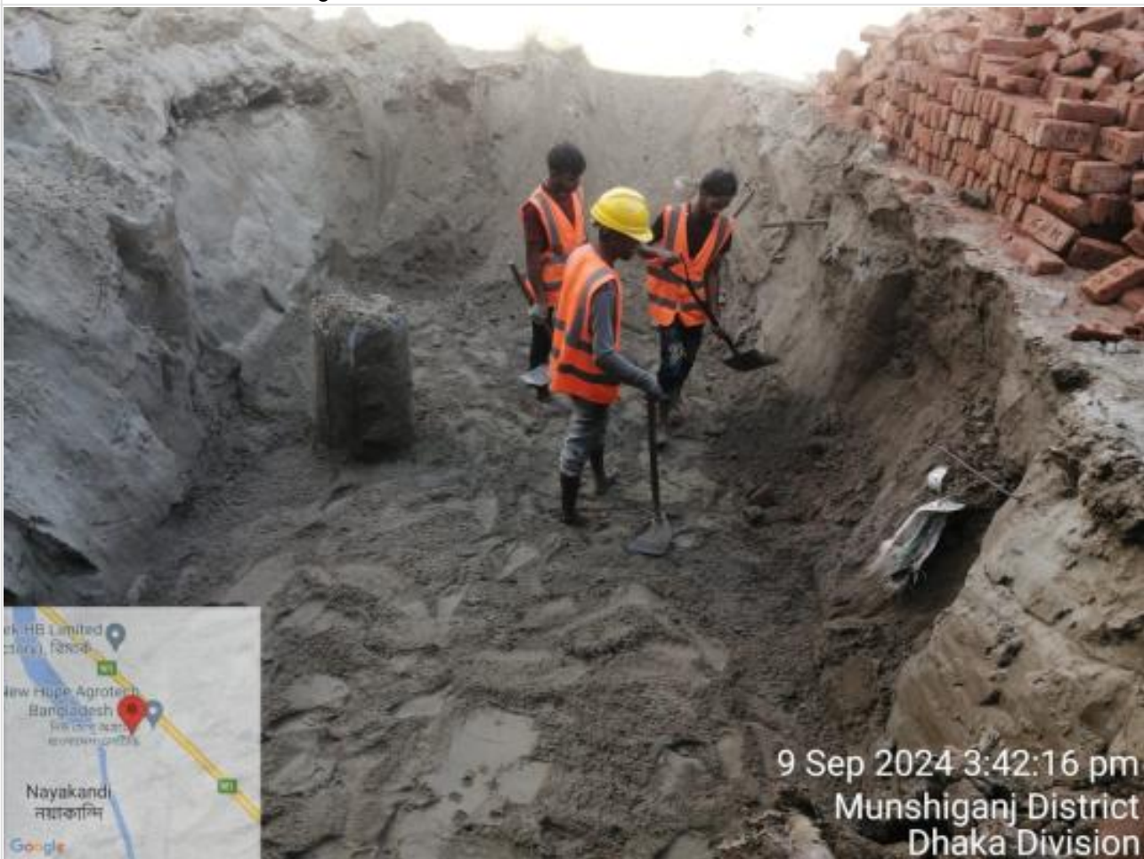
Excavation for pile mud tank on 09-09-24
