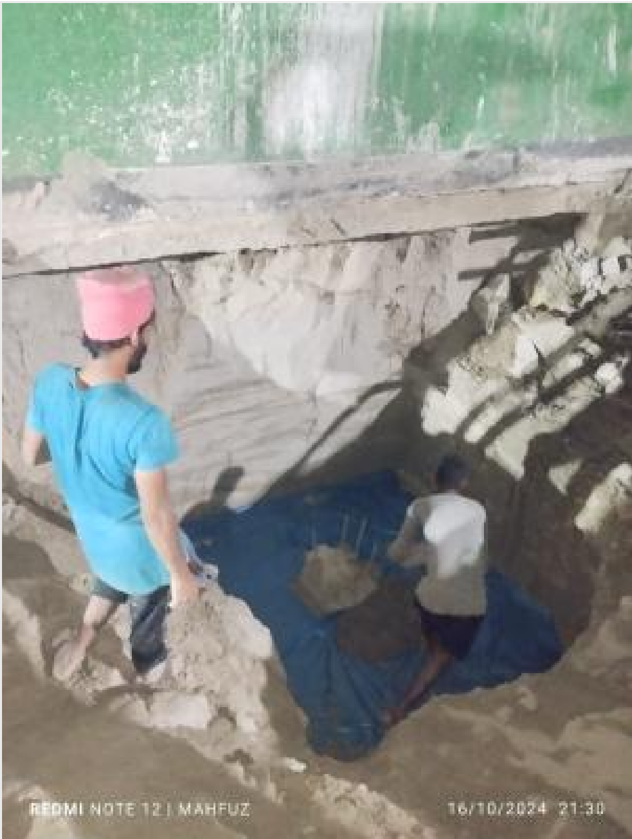
Pile Cap Lean concreting on 16-10-24
