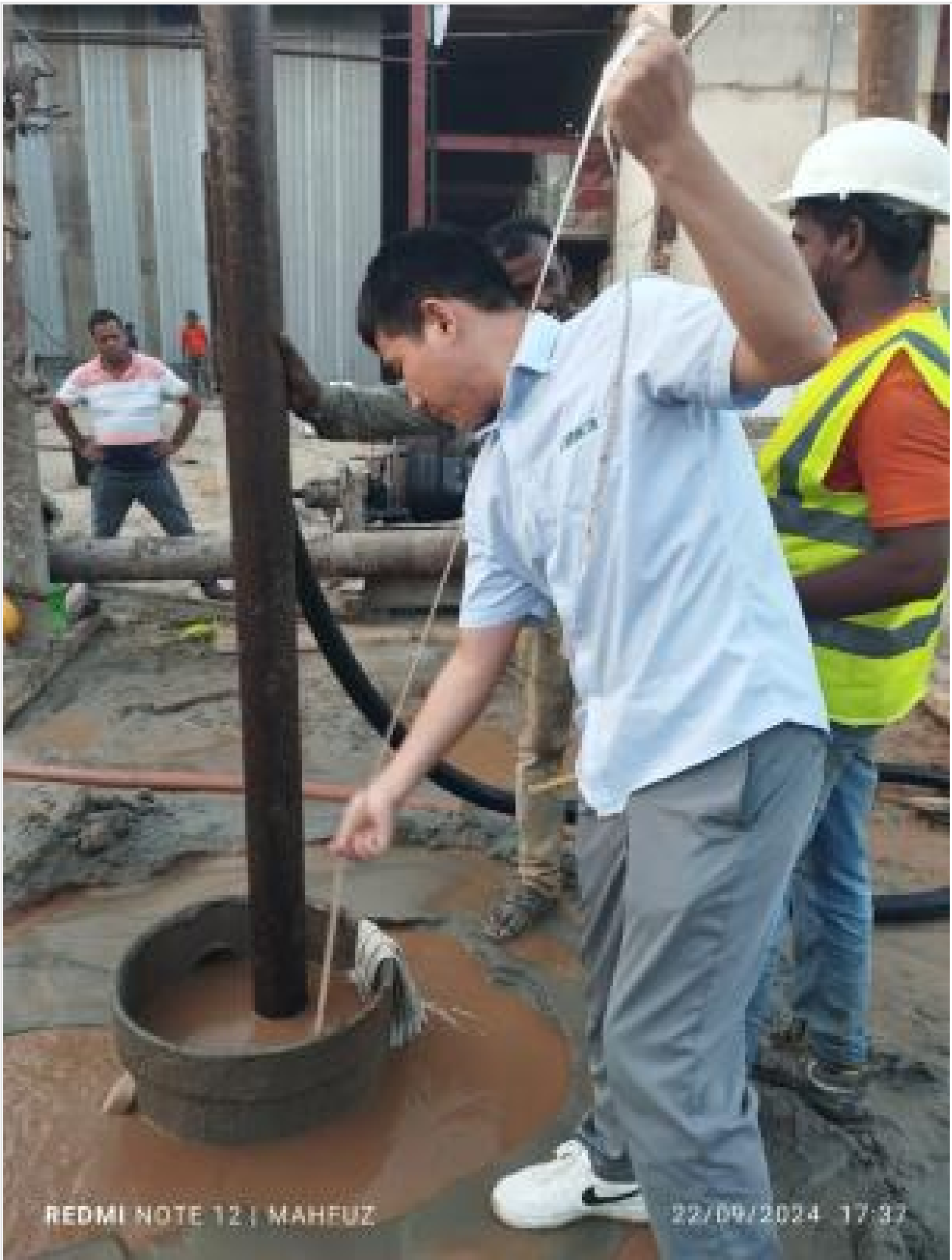
Pile boring length checking on 22-09-24
