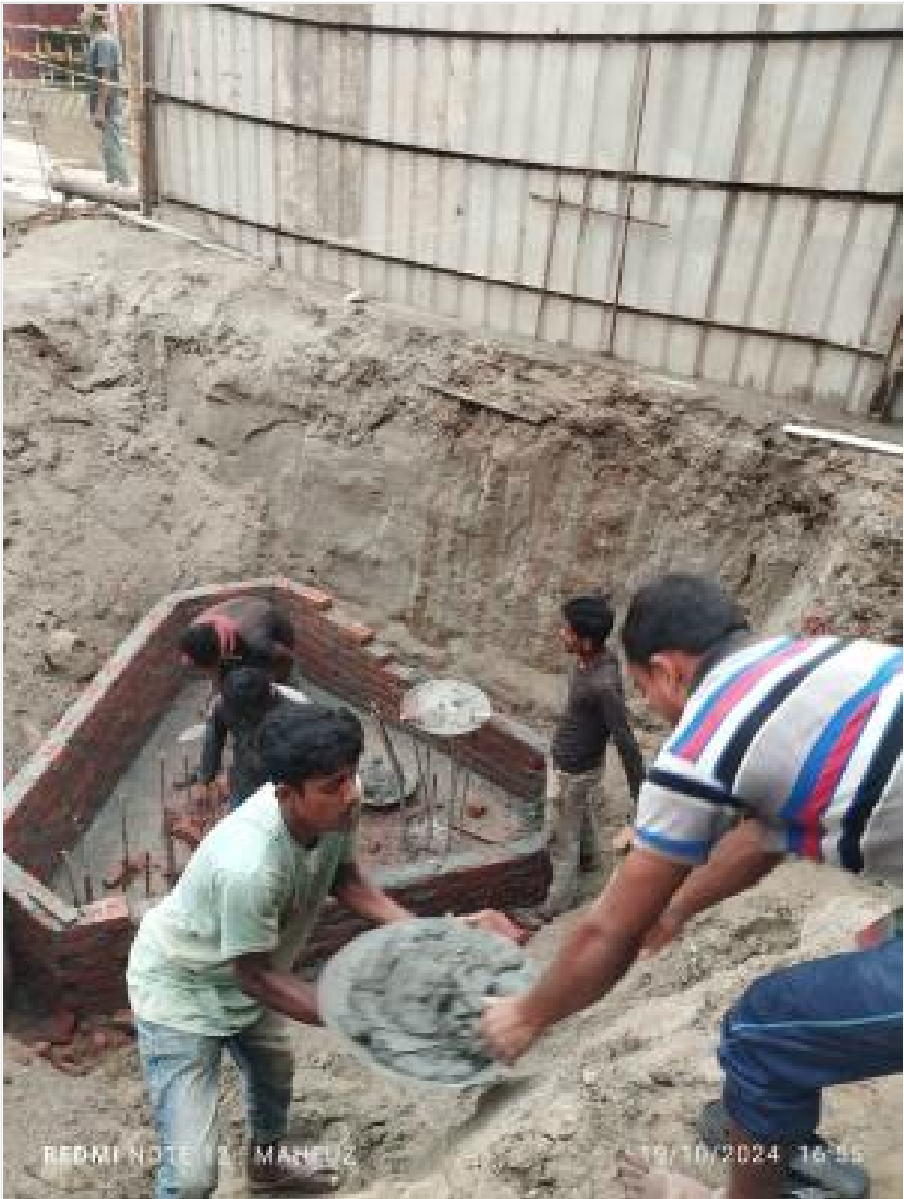
Pile Cap Brick Shuttering on 19-10-24
