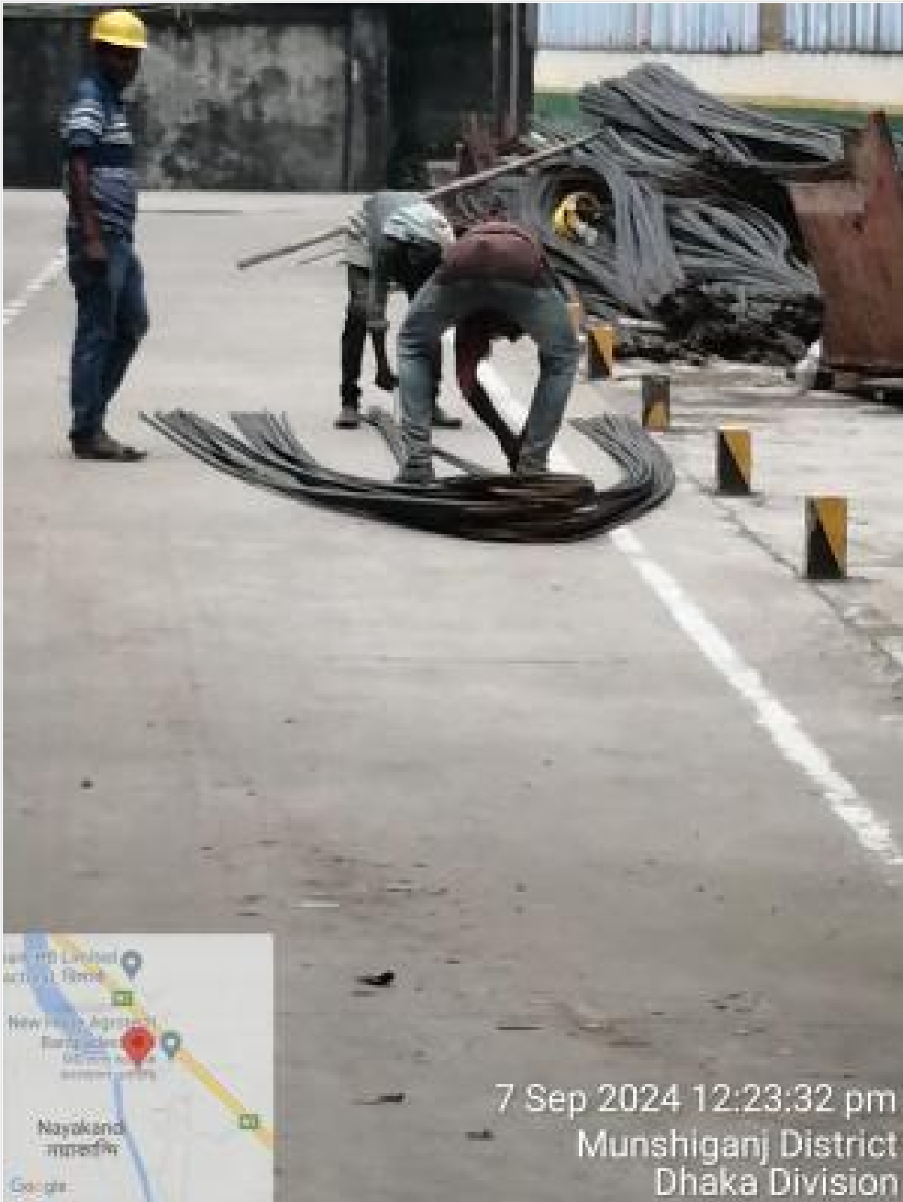
Pile Re-bar work on 07-09-24
