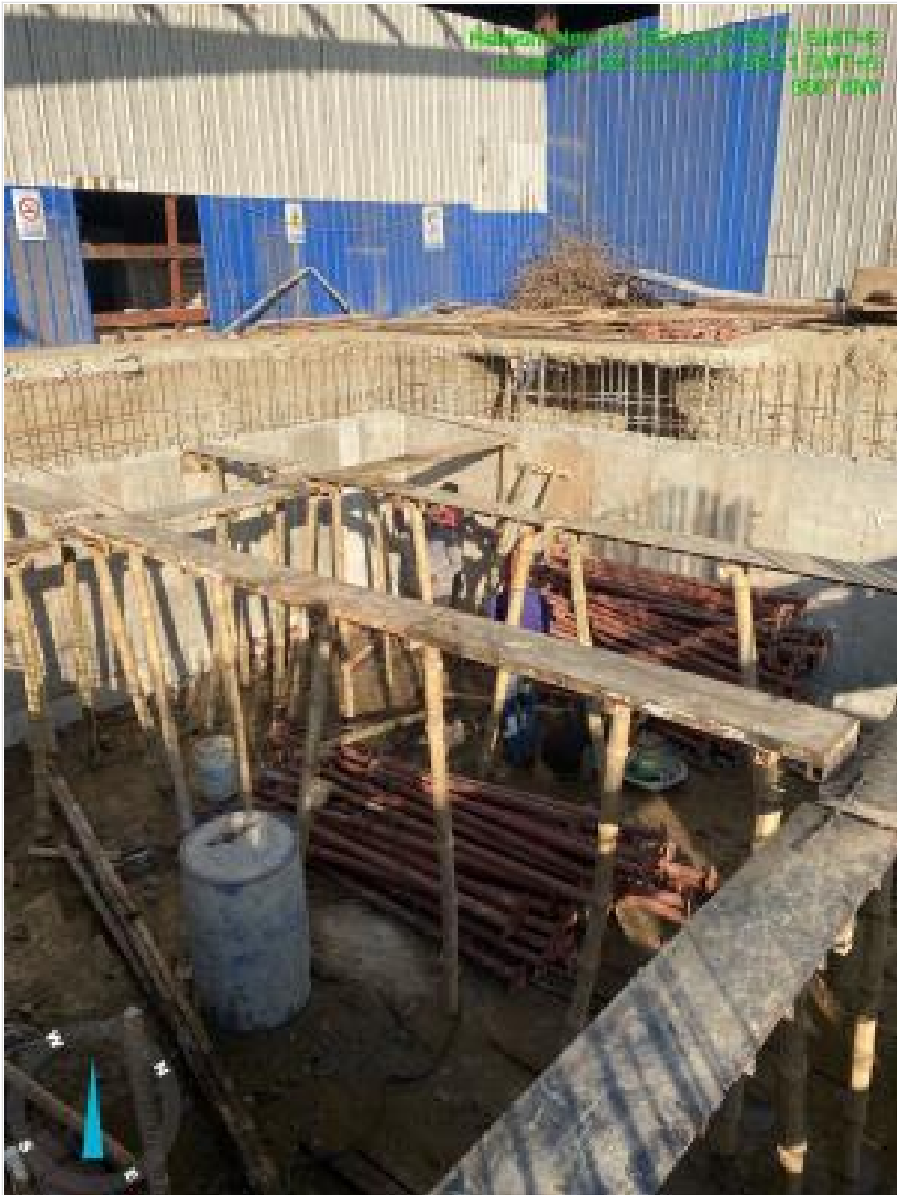
Tank slab shuttering on 19-11-24
