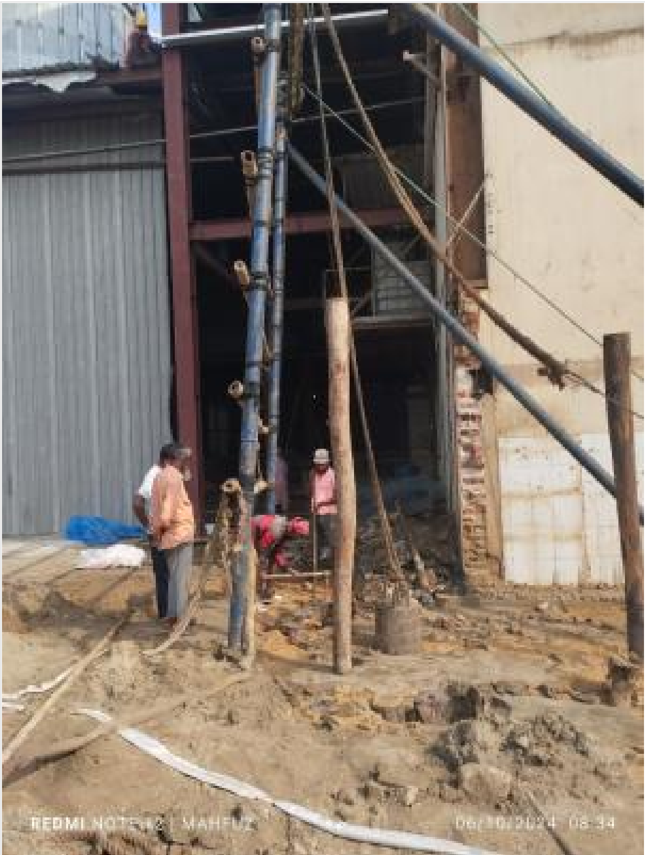
Wooden shore pile driving on 06-10-24
