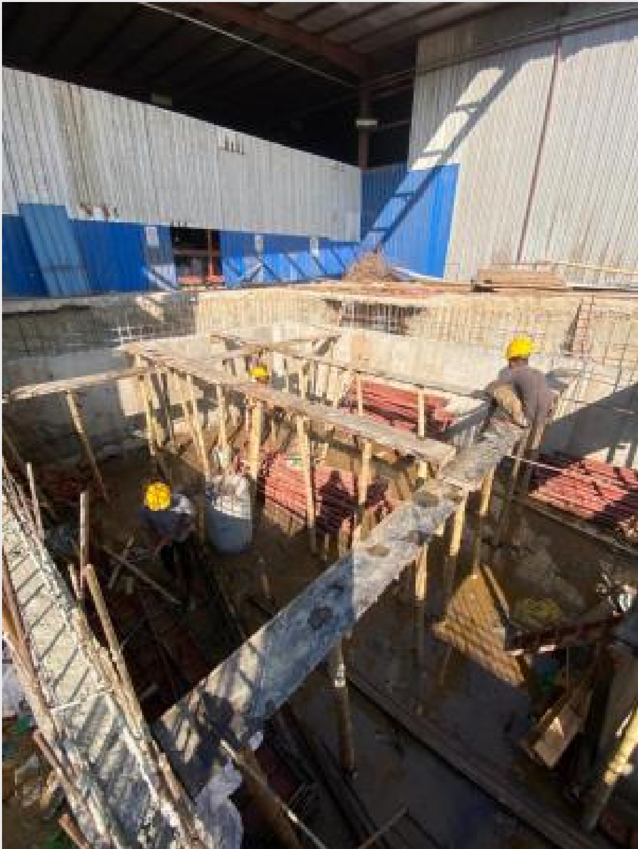
Tank slab shuttering on 20-11-24
