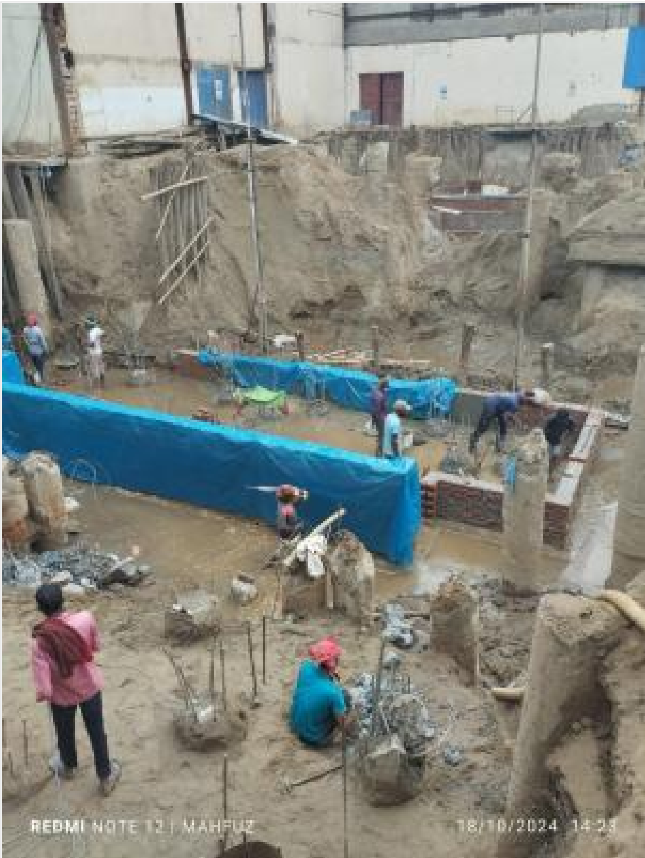
Pile head breaking on 18-10-24
