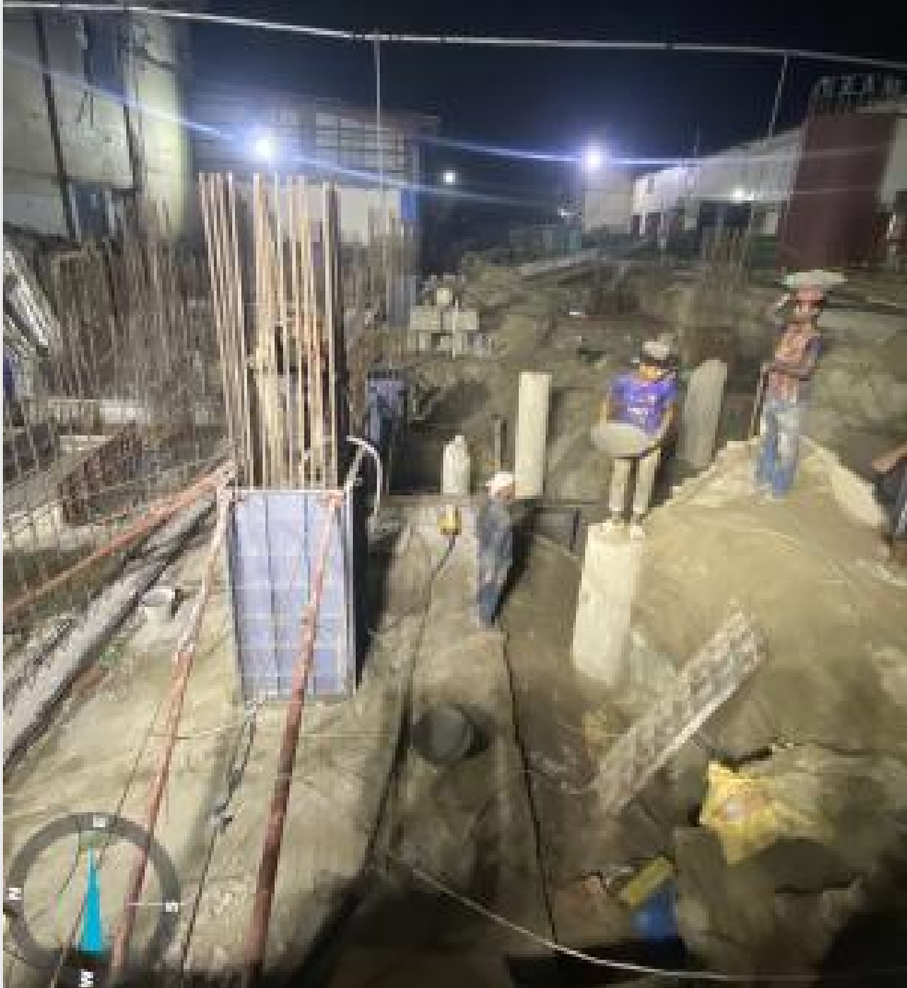
Column concreting on 04-11-24
