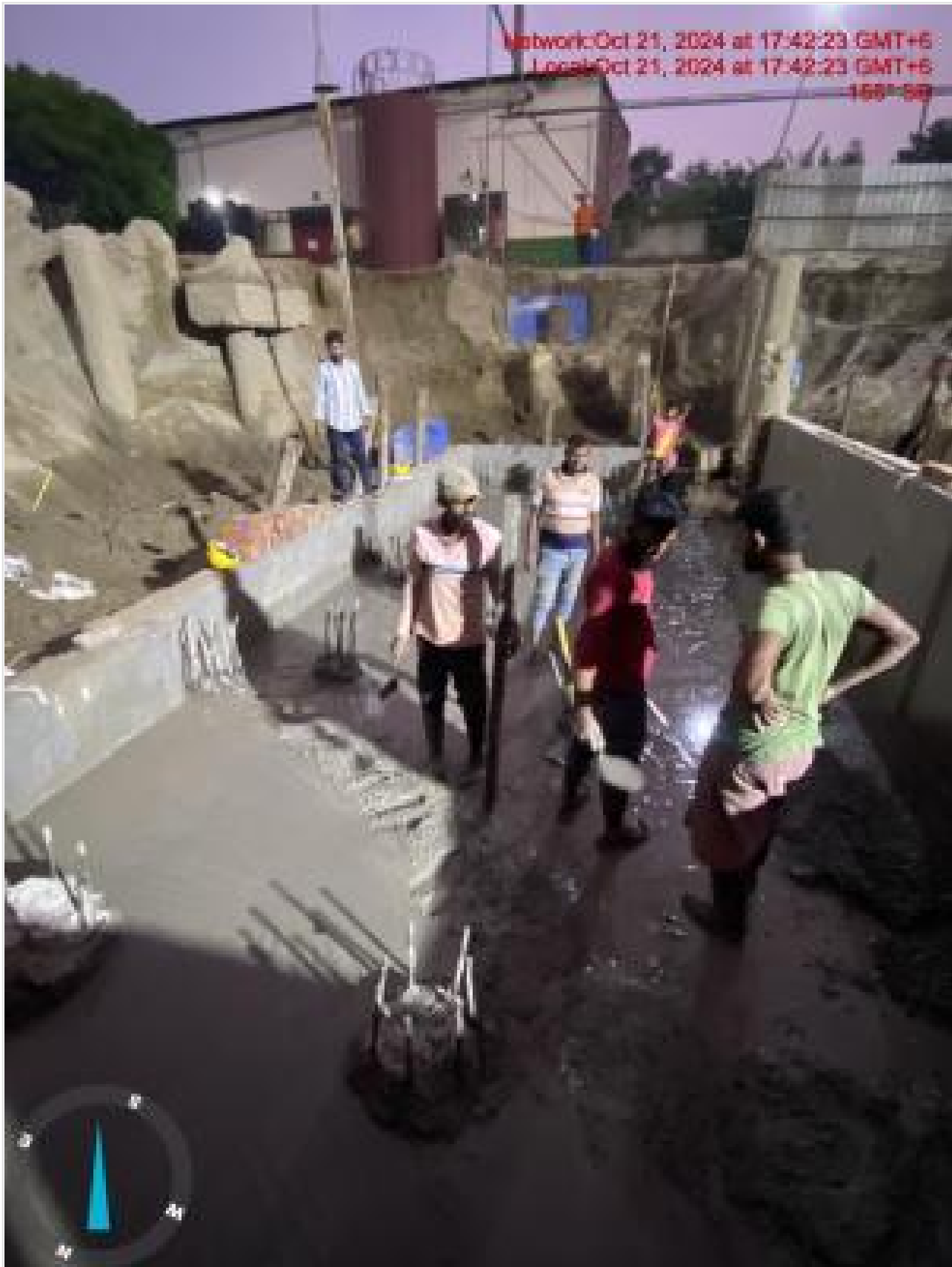
Pile cap lean concreting on 21-10-24
