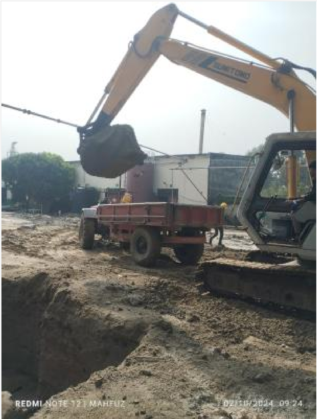
Earth excavation on 02-10-24
