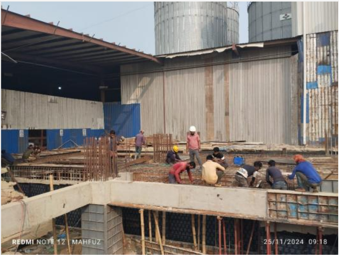
Tank Slab Re-bar work on 25-11-24
