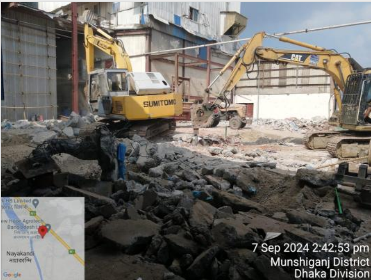
Floor and Foundation Removal on 07-09-24
