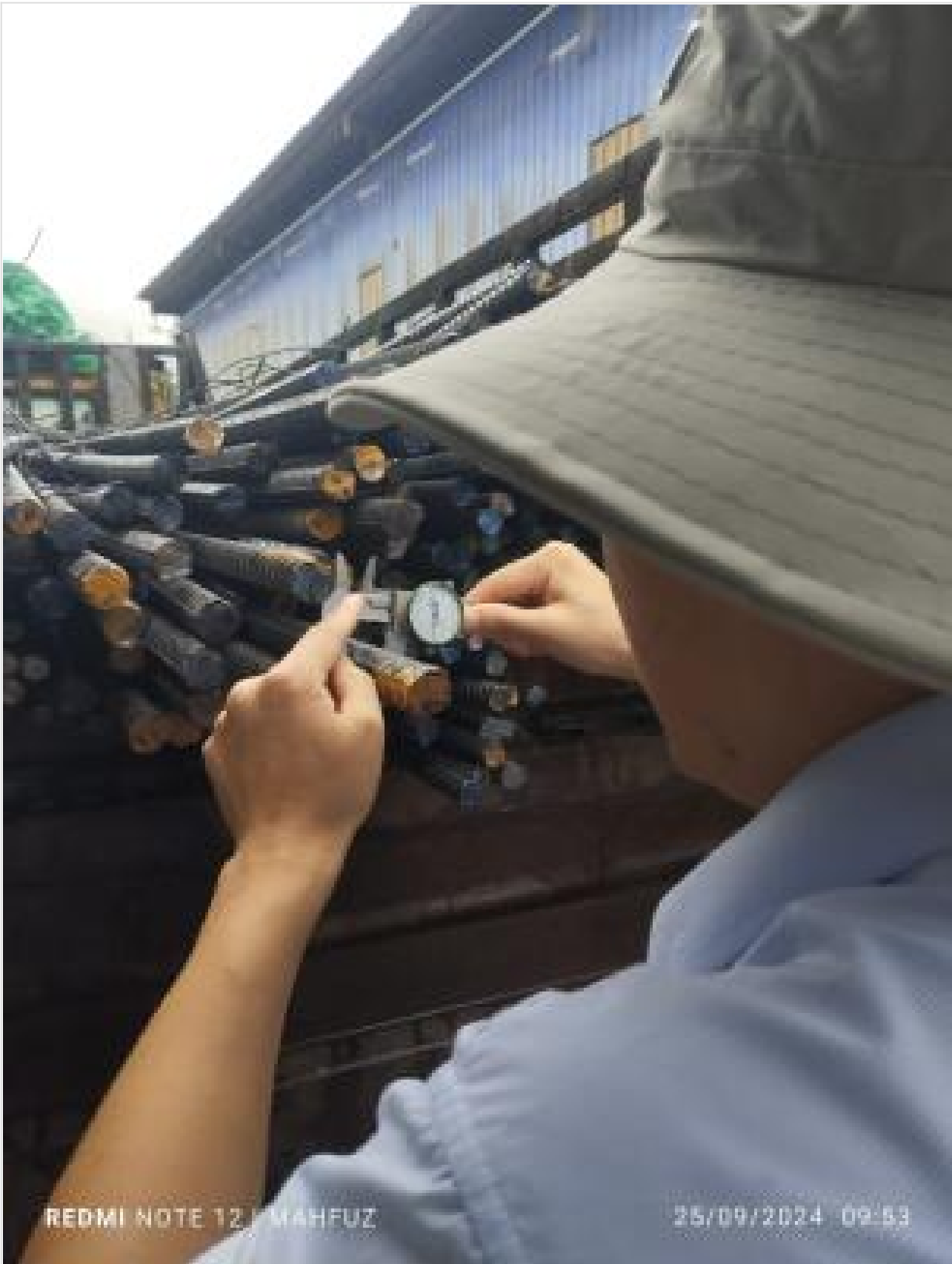
Pile cap re-bar dia checking on 25-09-24
