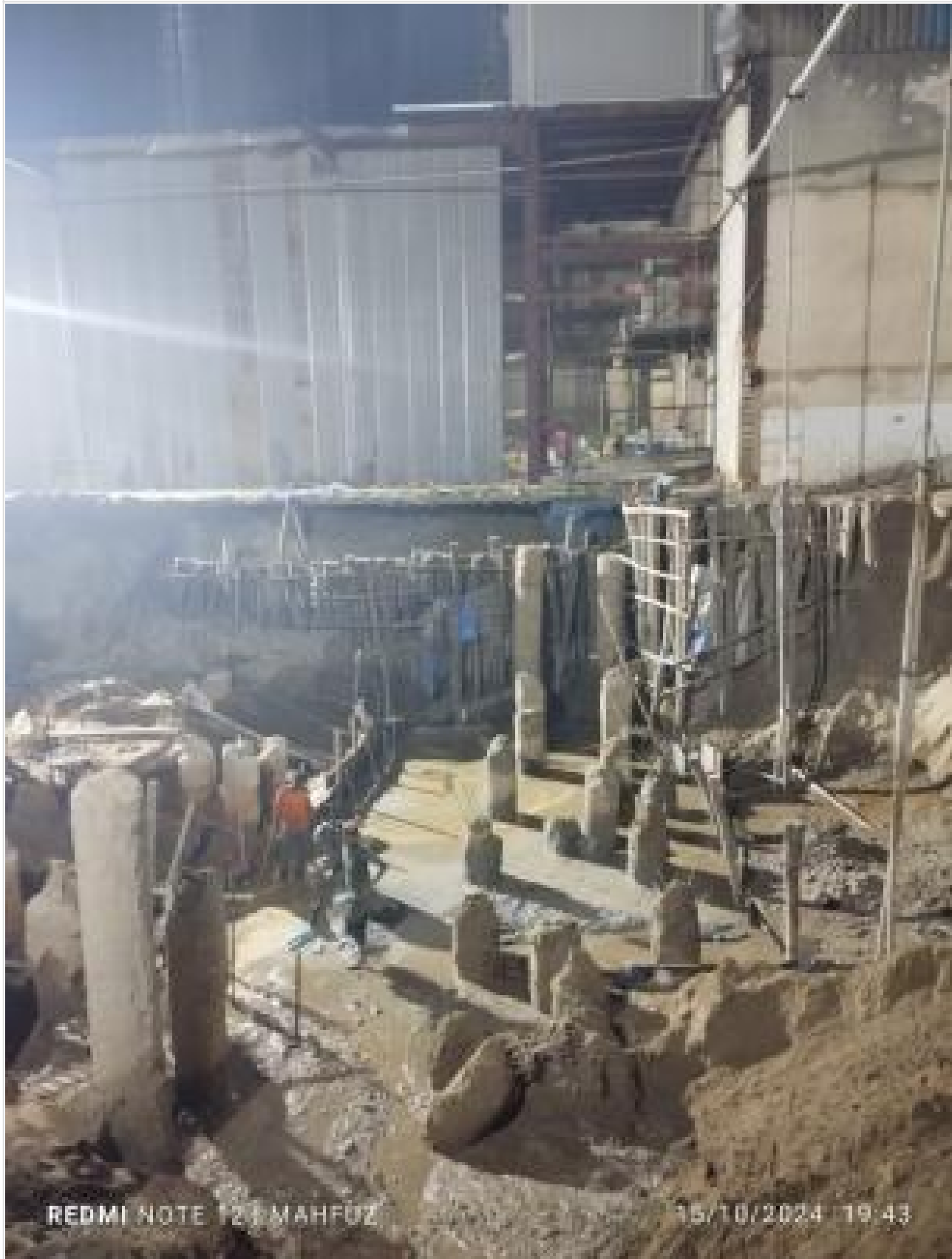
CC at level -5200 finished on 15-10-24
