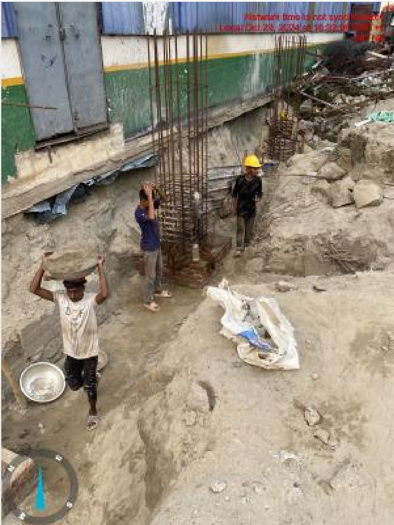
Earth excavation on 29-10-24
