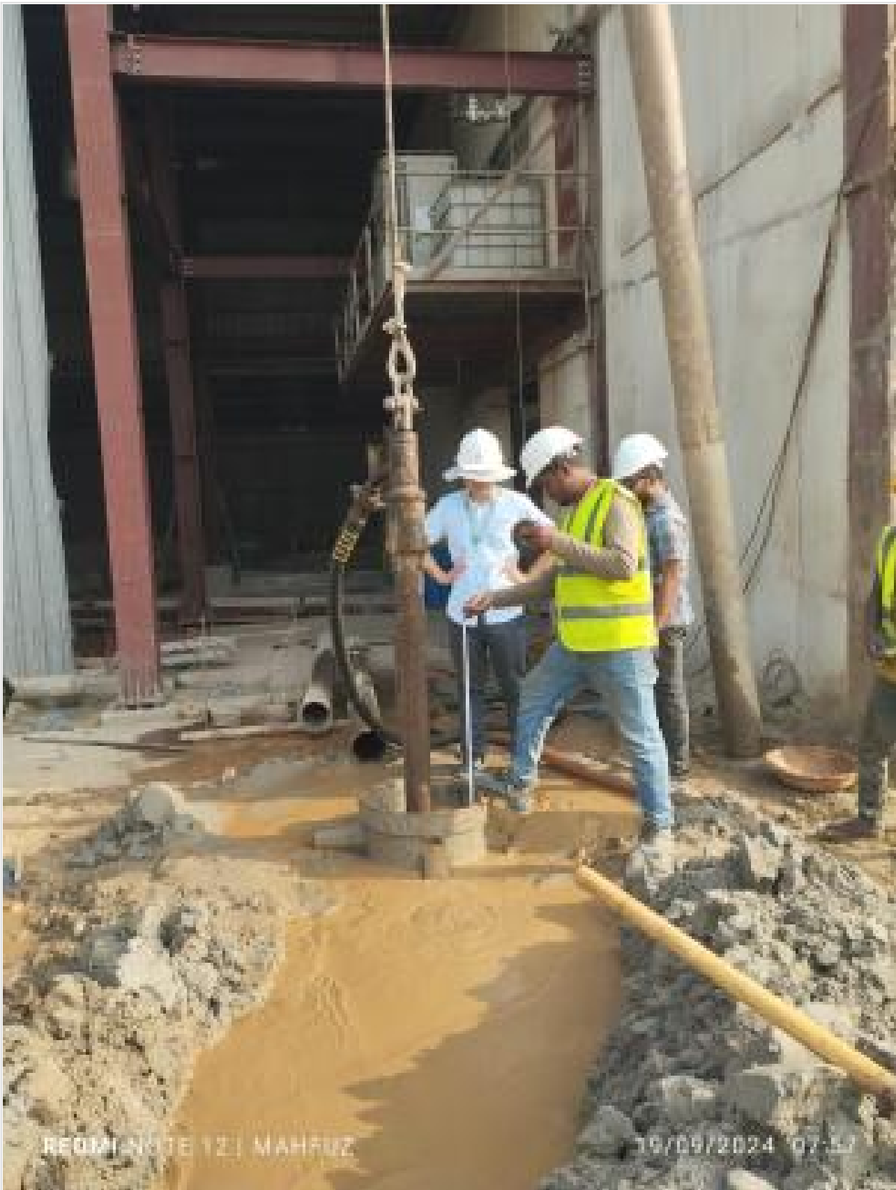
Pile boring length checking on 19-09-24
