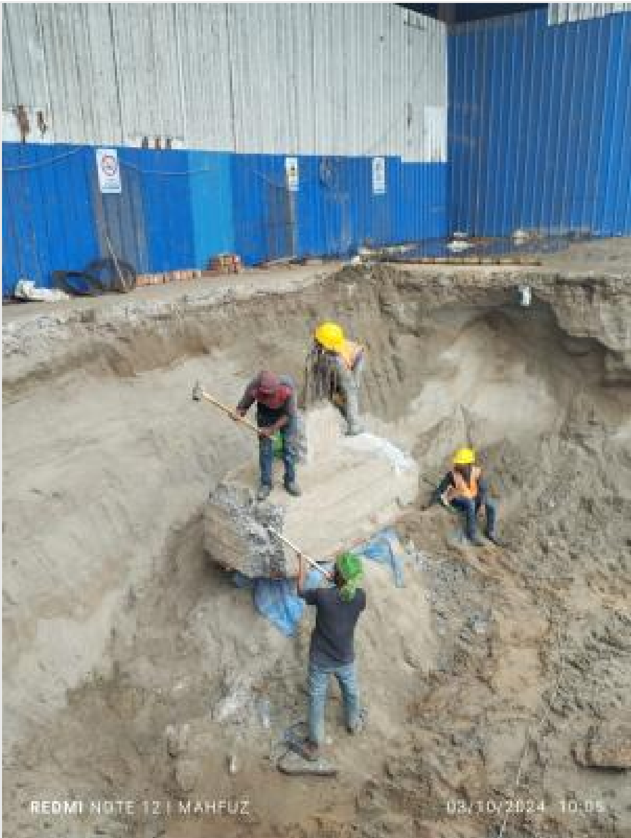
Obstacle RCC dismantling on 03-10-24
