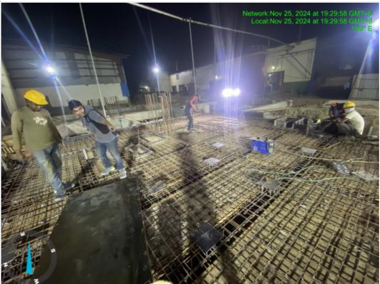
Embedded steel part fixing on 25-11-24
