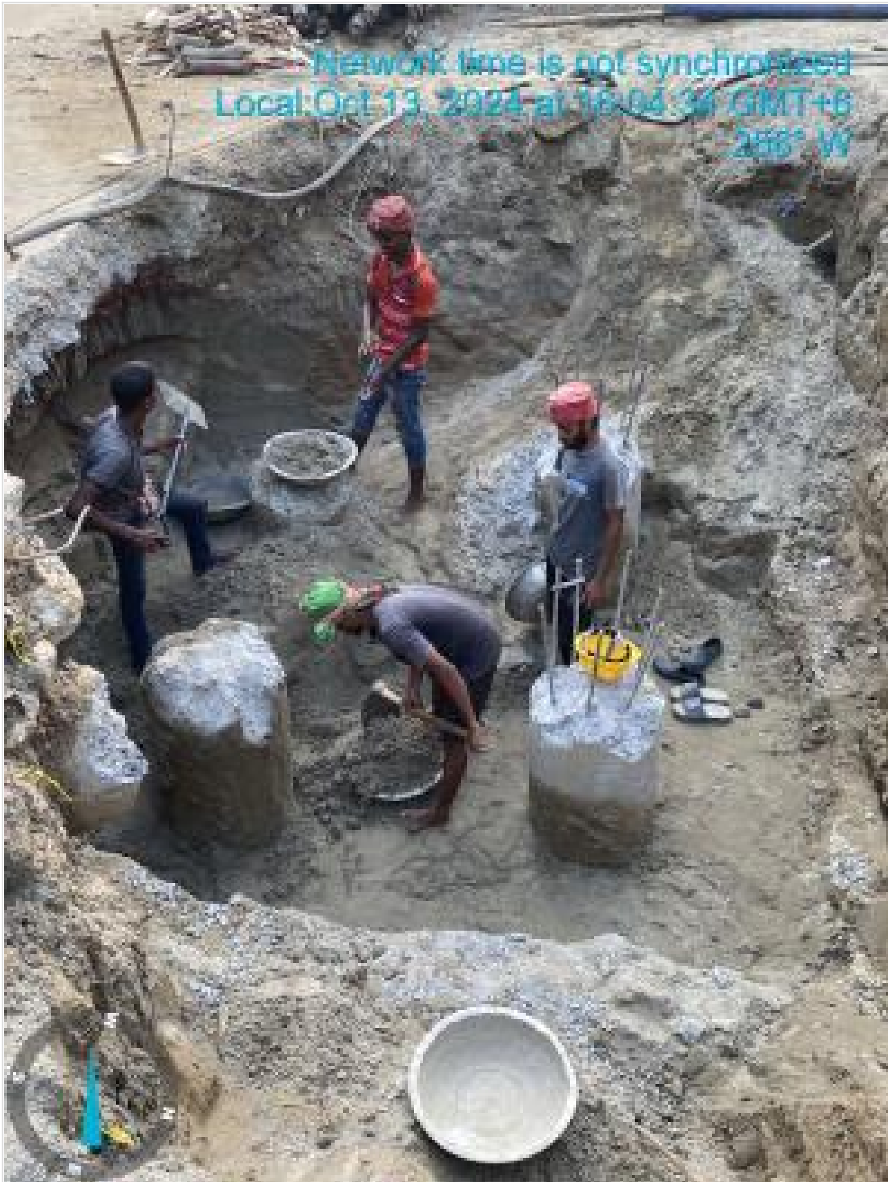
Earth excavation manually on 13-10-24
