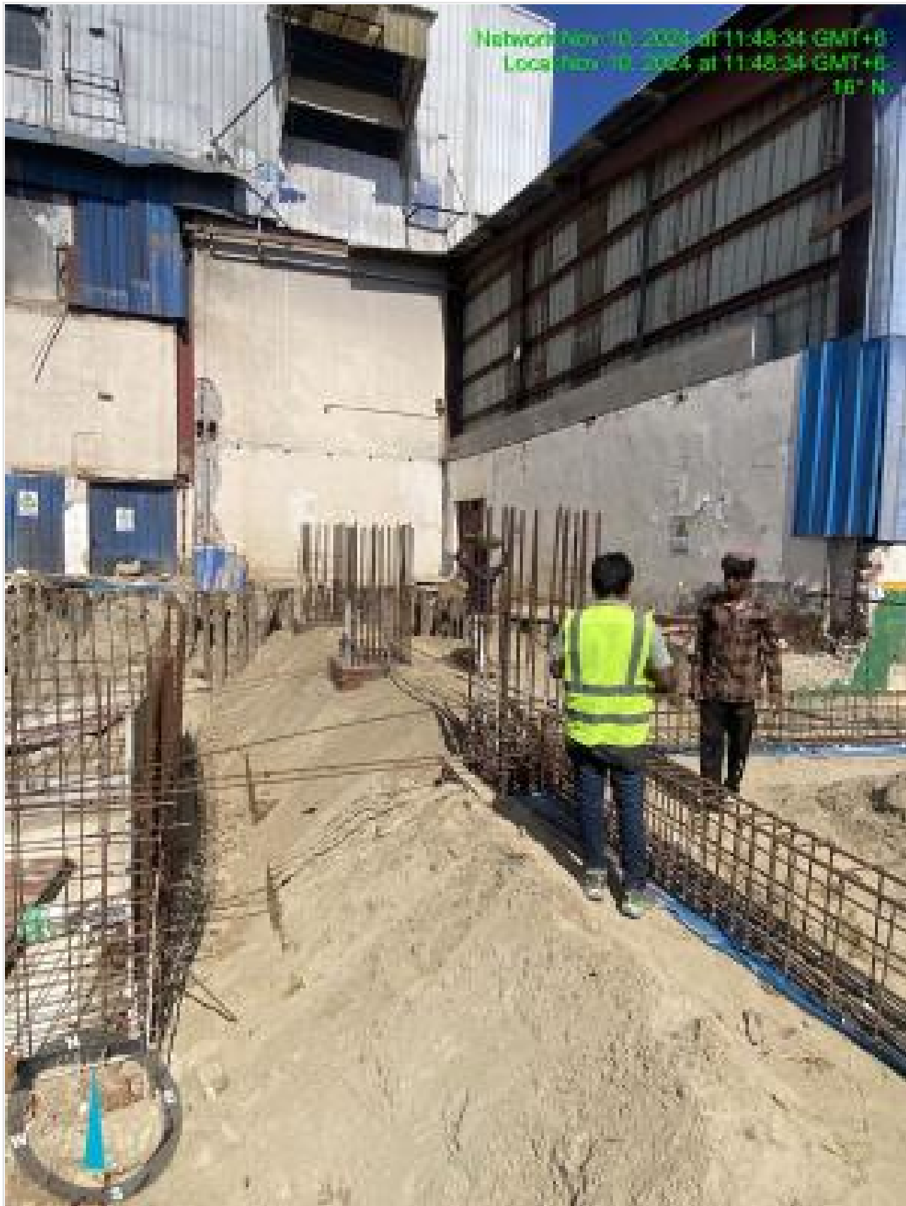
Foundation beam rebar work on 10-11-24
