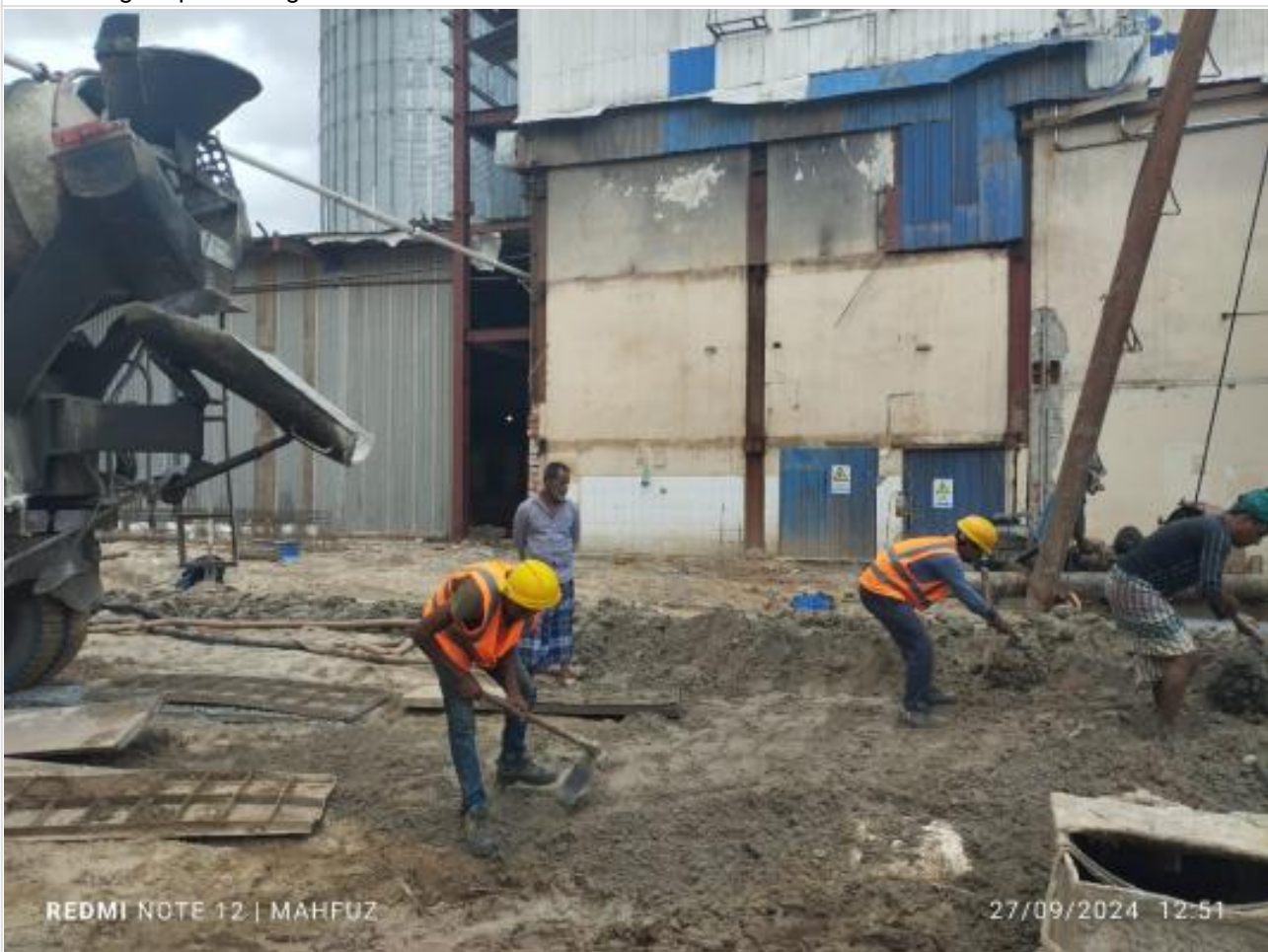
Making road for reading concrete truck on 27-09-24
