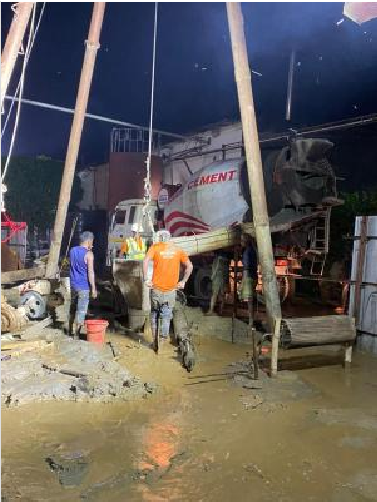
Pile concreting on 22-09-24
