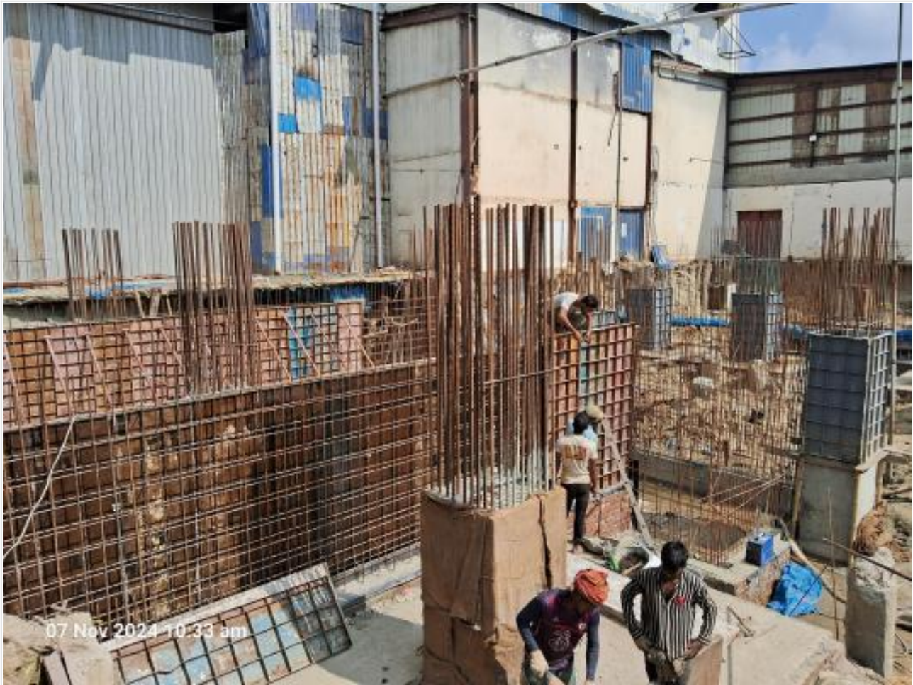
Wall shuttering on 07-11-24
