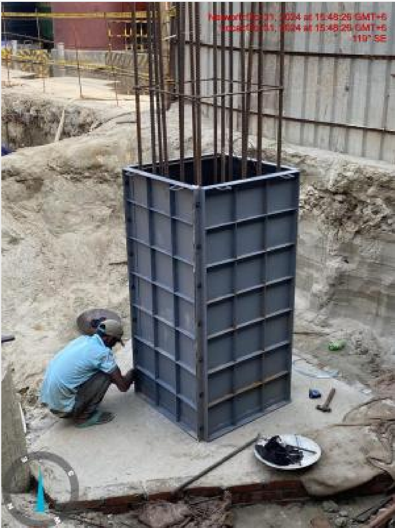
Column Shuttering on 31-10-24
