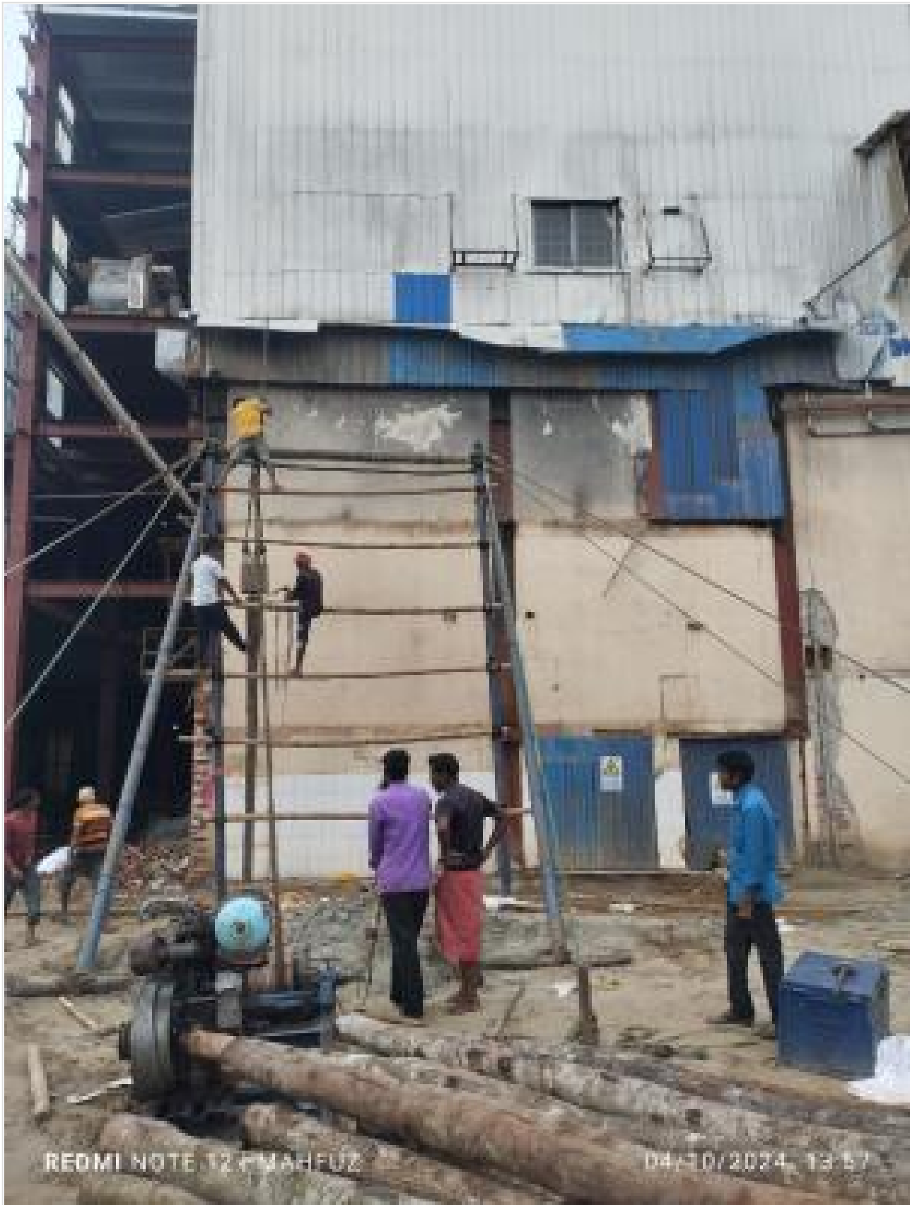
Wooden pile driving on 04-10-24
