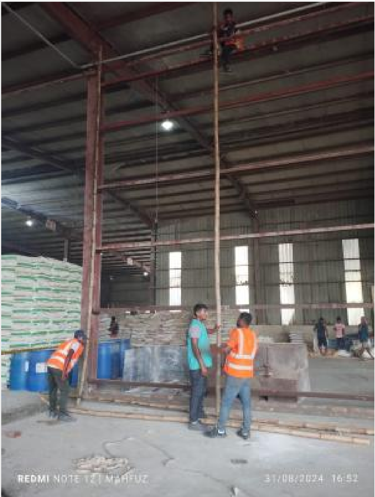
Fencing framing on 31-08-24
