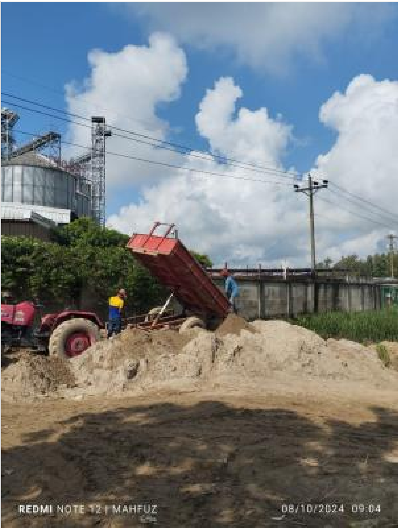
Excavated earth dumping on 08-10-24
