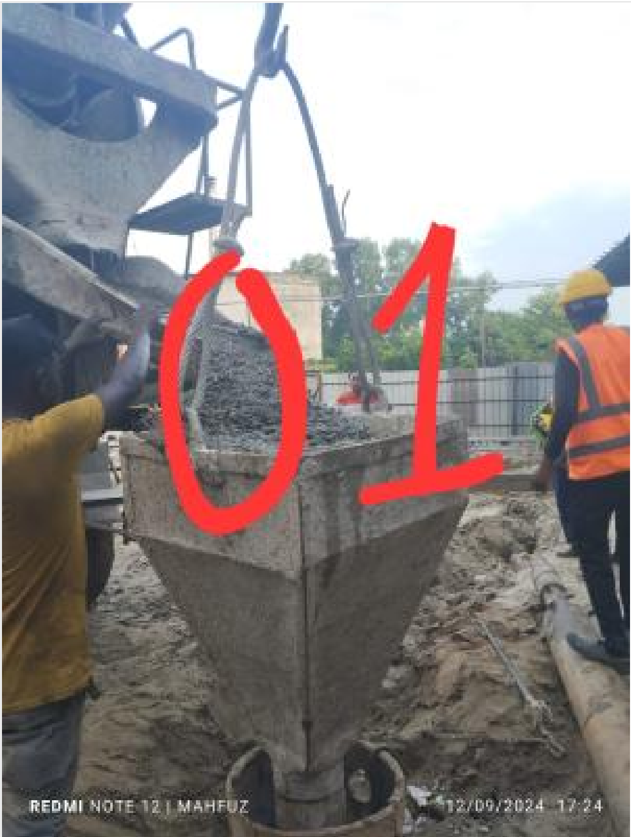
Pile concreting on 12-09-24
