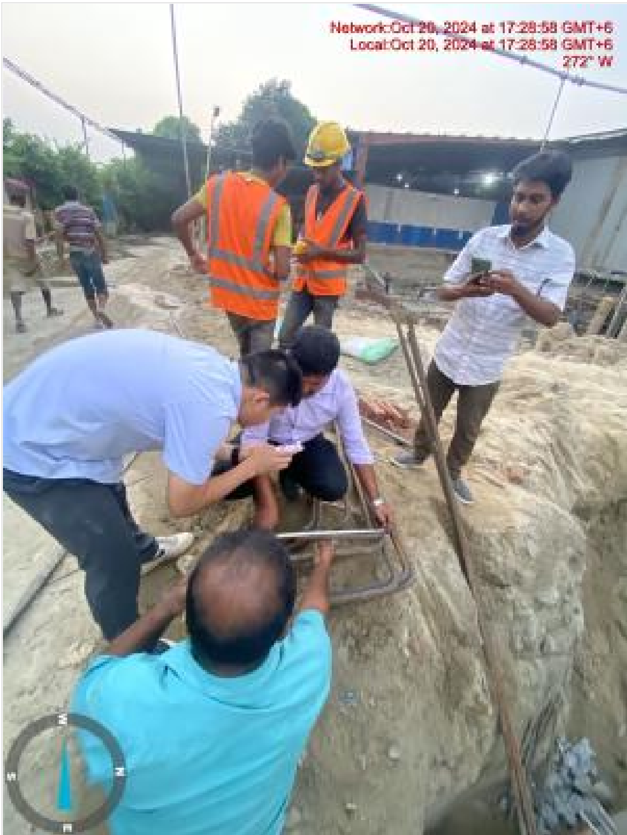
PIT (Pile Integrity) testing on 20-10-24
