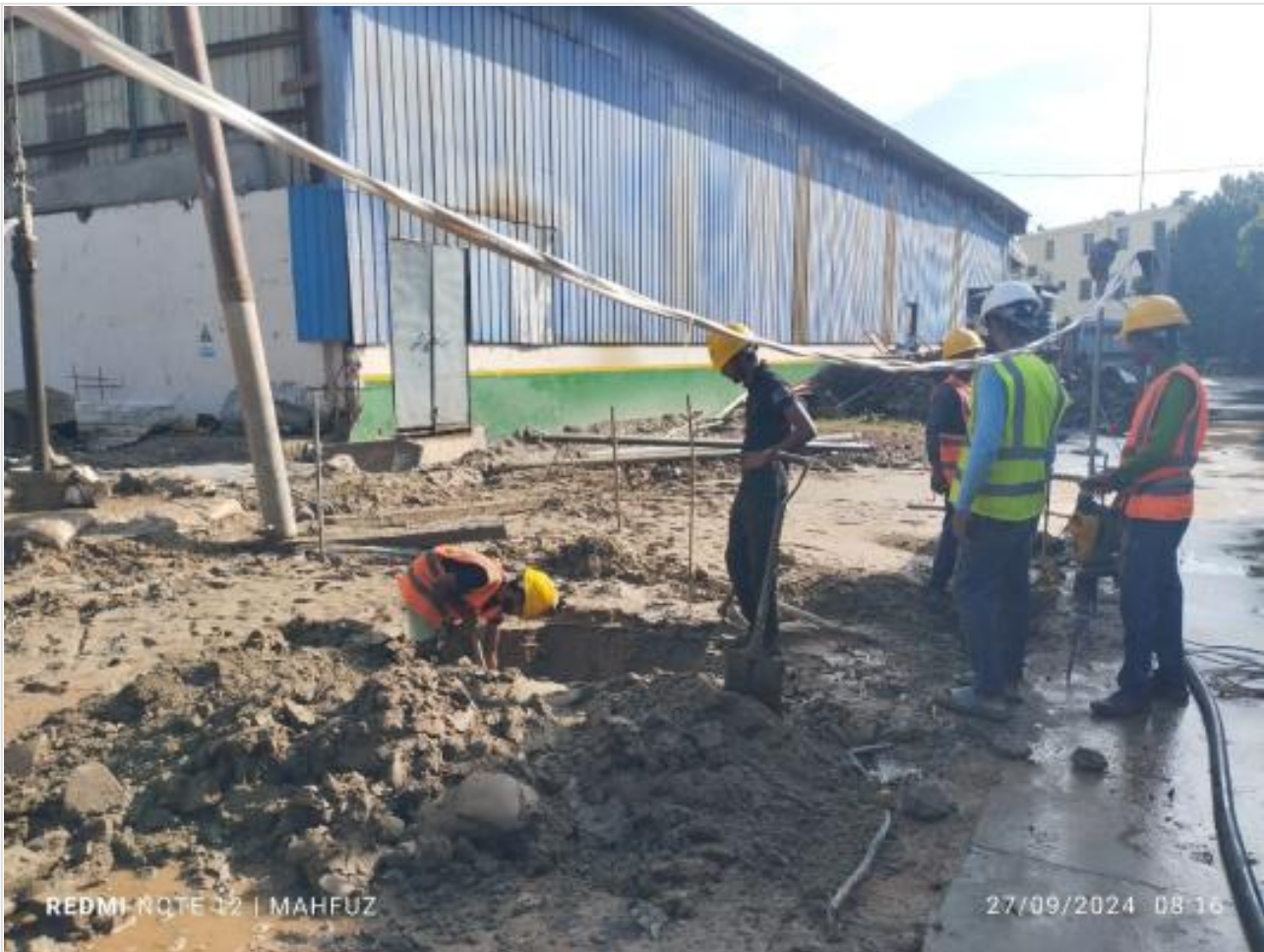
Excavating for pile boring obstacles on 27-09-24
