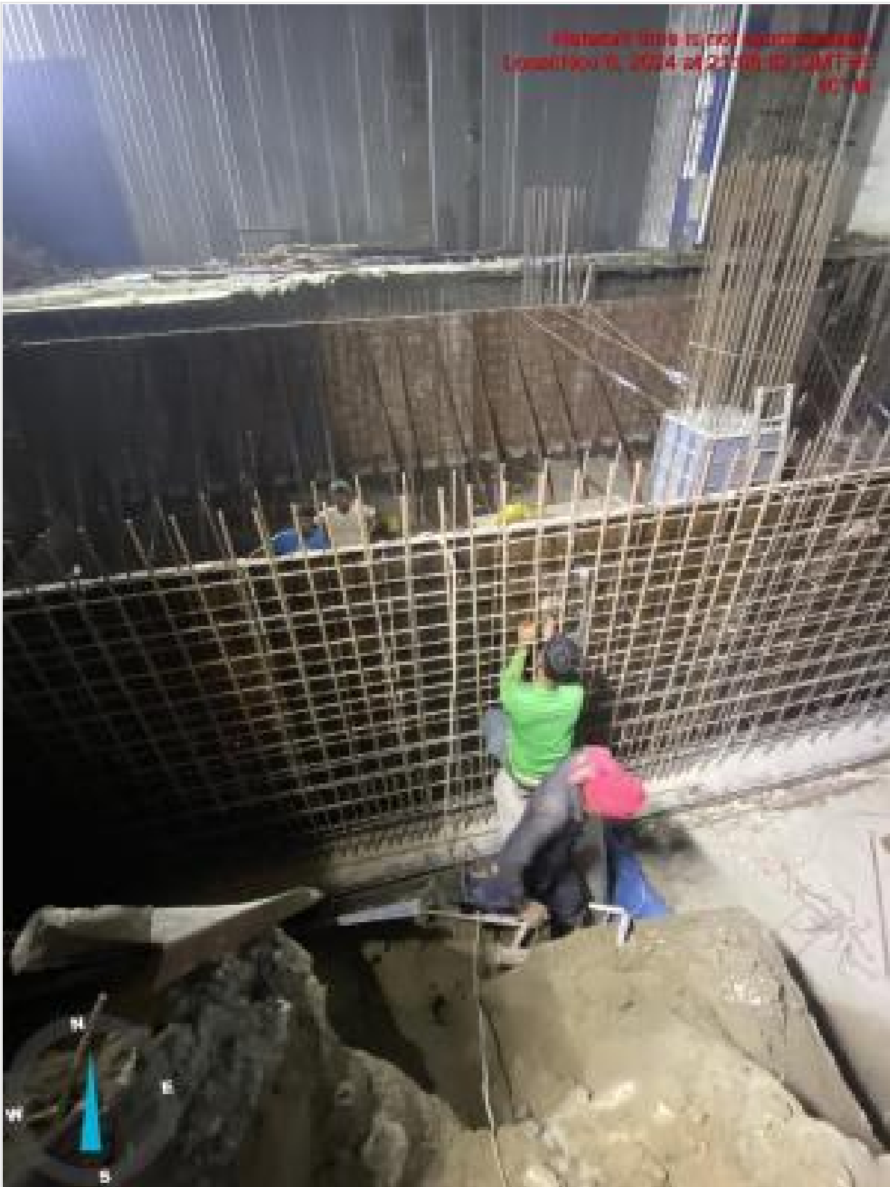
Wall shuttering on 06-11-24
