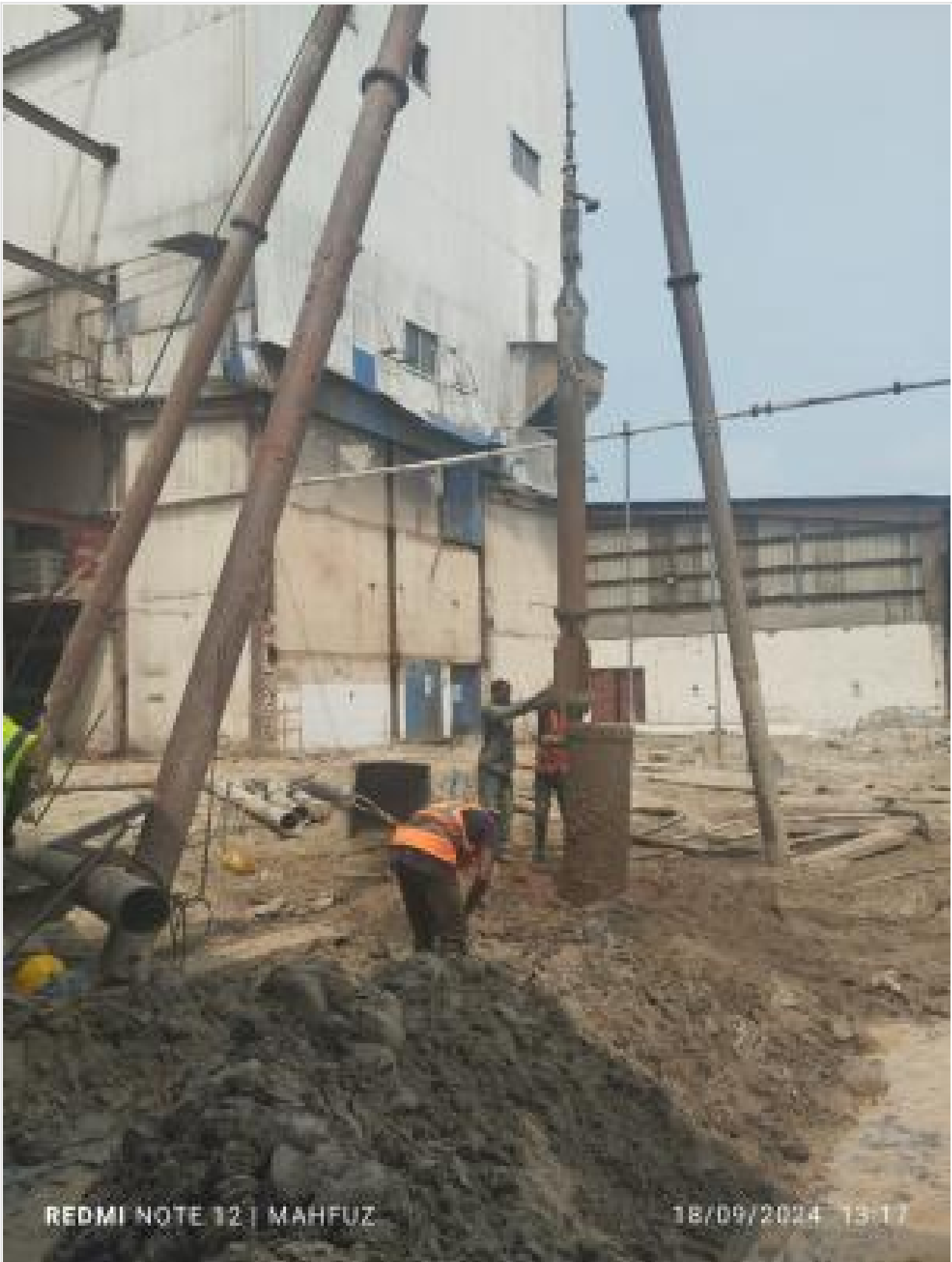
Pile reboring new location on 18-09-24
