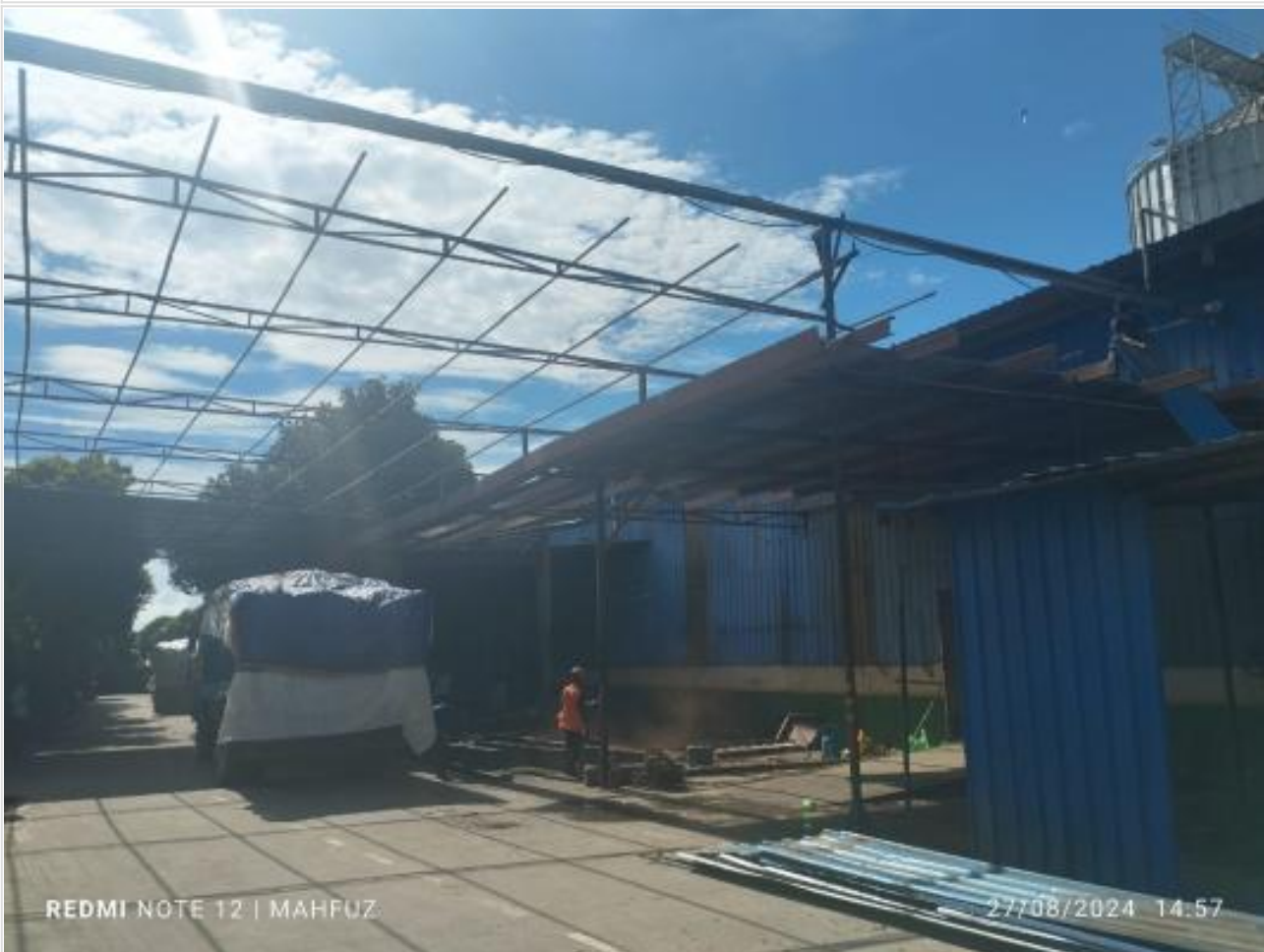
Workshop Sheet Removing on 27-08-24
