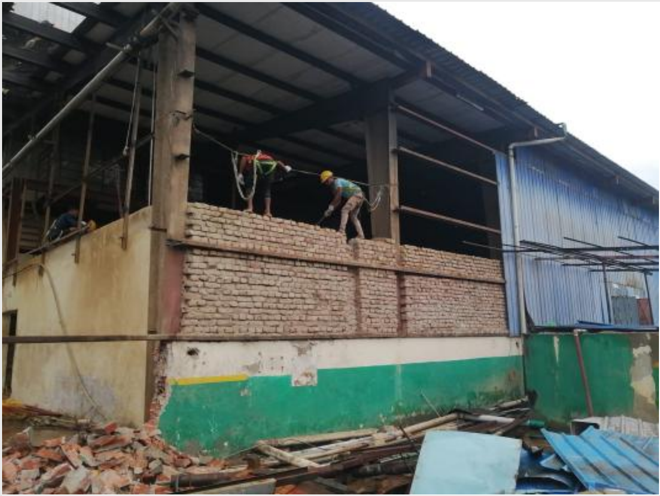
Brick wall dismantling on 03-09-24
