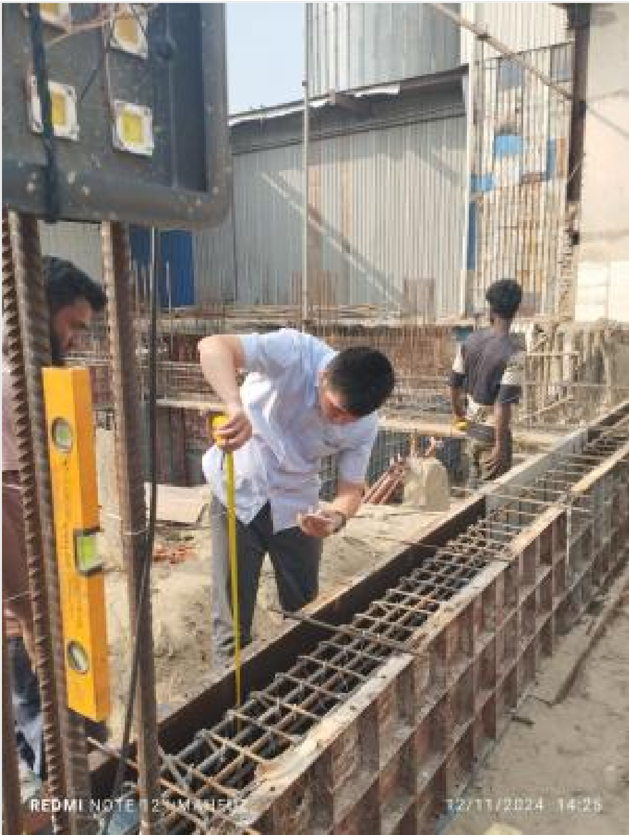
Foundation beam inspection before concrete on 12-11-24
