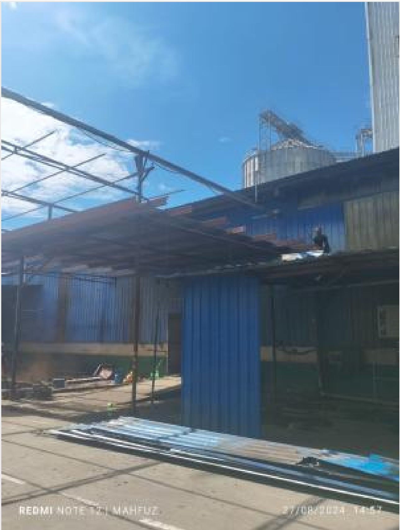
Workshop Sheet Removing on 27-08-24
