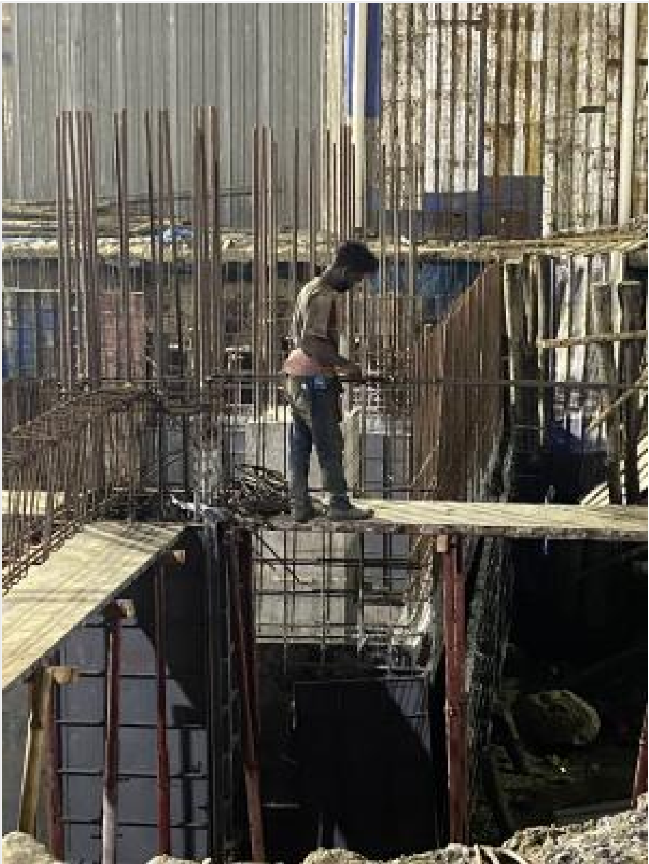
Foundation beam rebar work on 11-11-24
