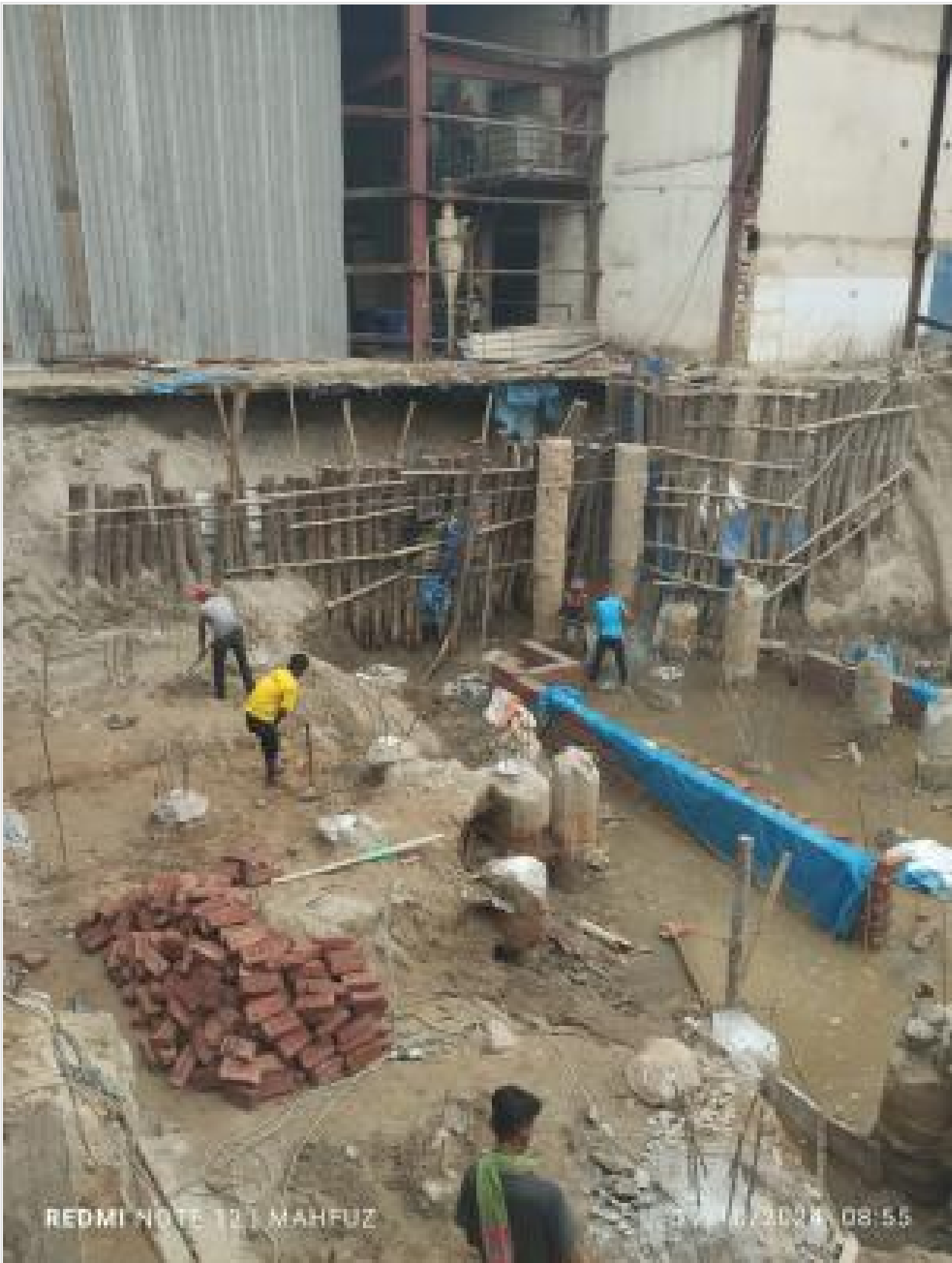
Pile head breaking on 17-10-24
