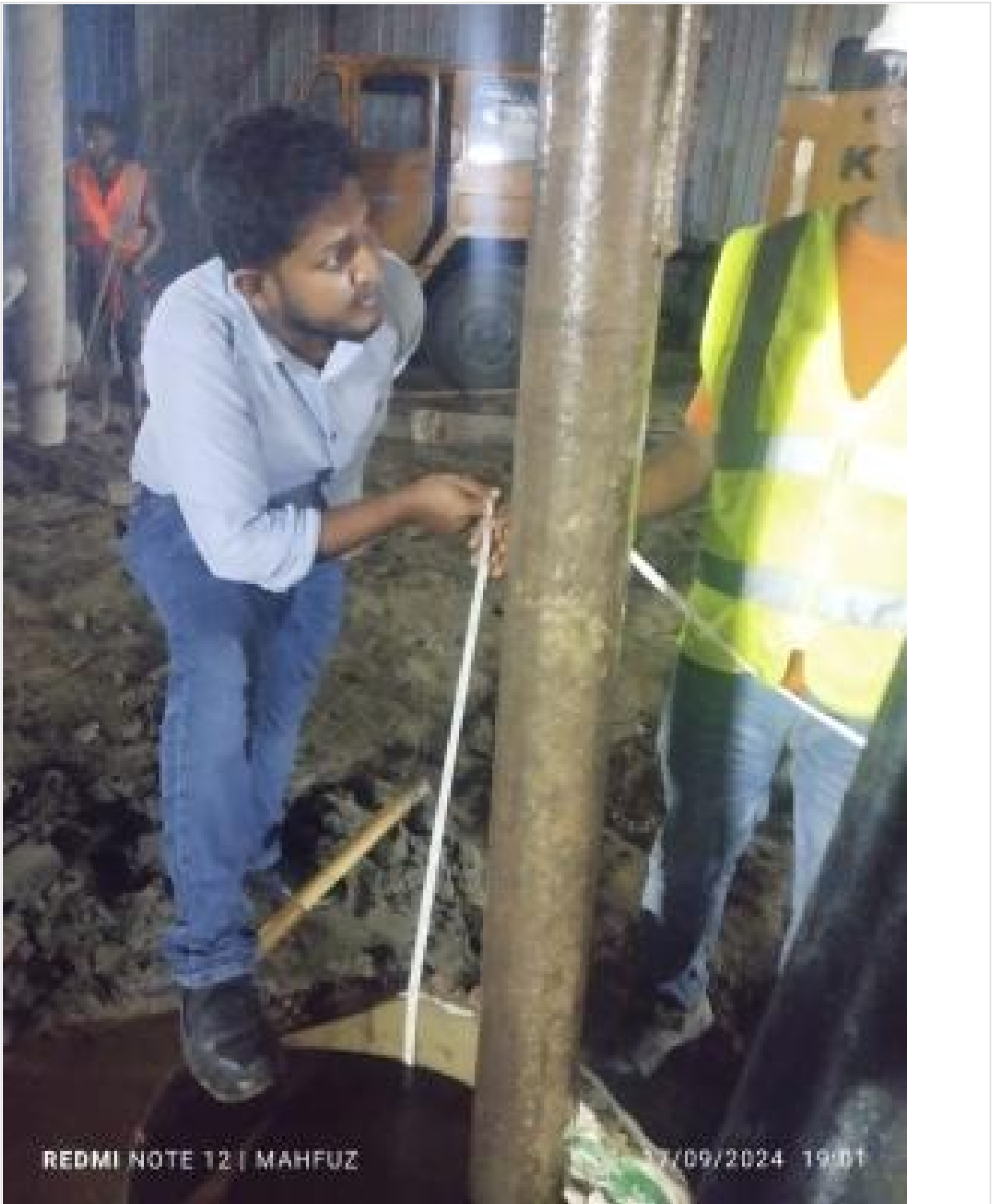
Pile boring length checking on 17-09-24
