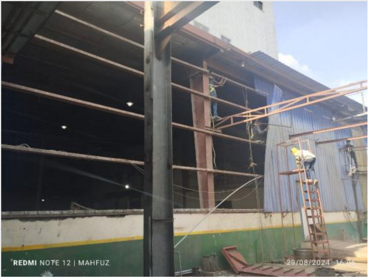
Sheet removing on 29-08-24
