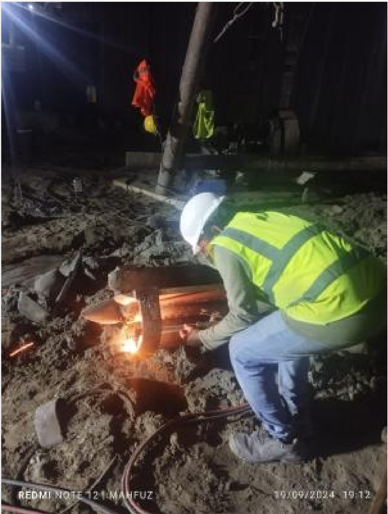
Pile boring chisel repairing on 19-09-24
