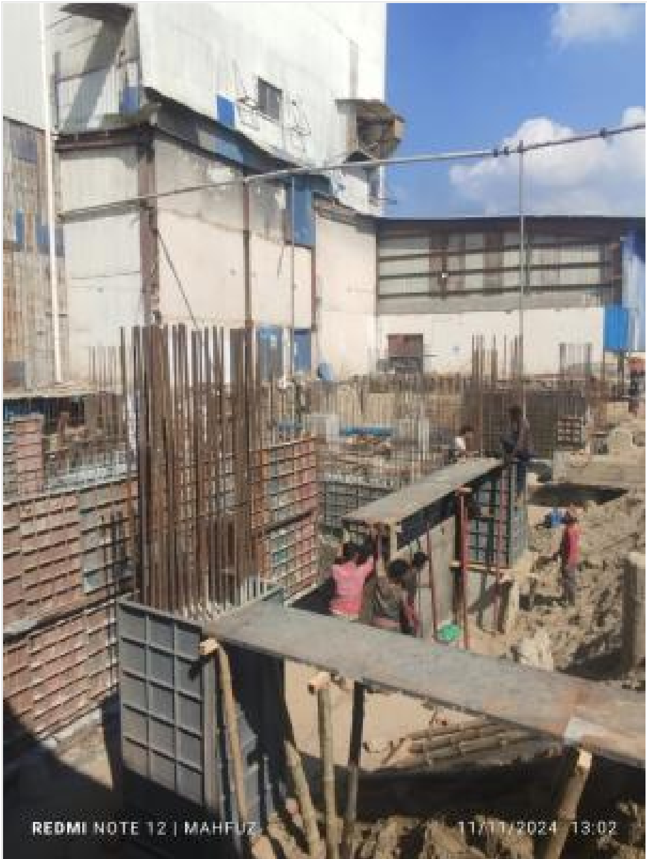
Foundation beam shuttering on 11-11-24
