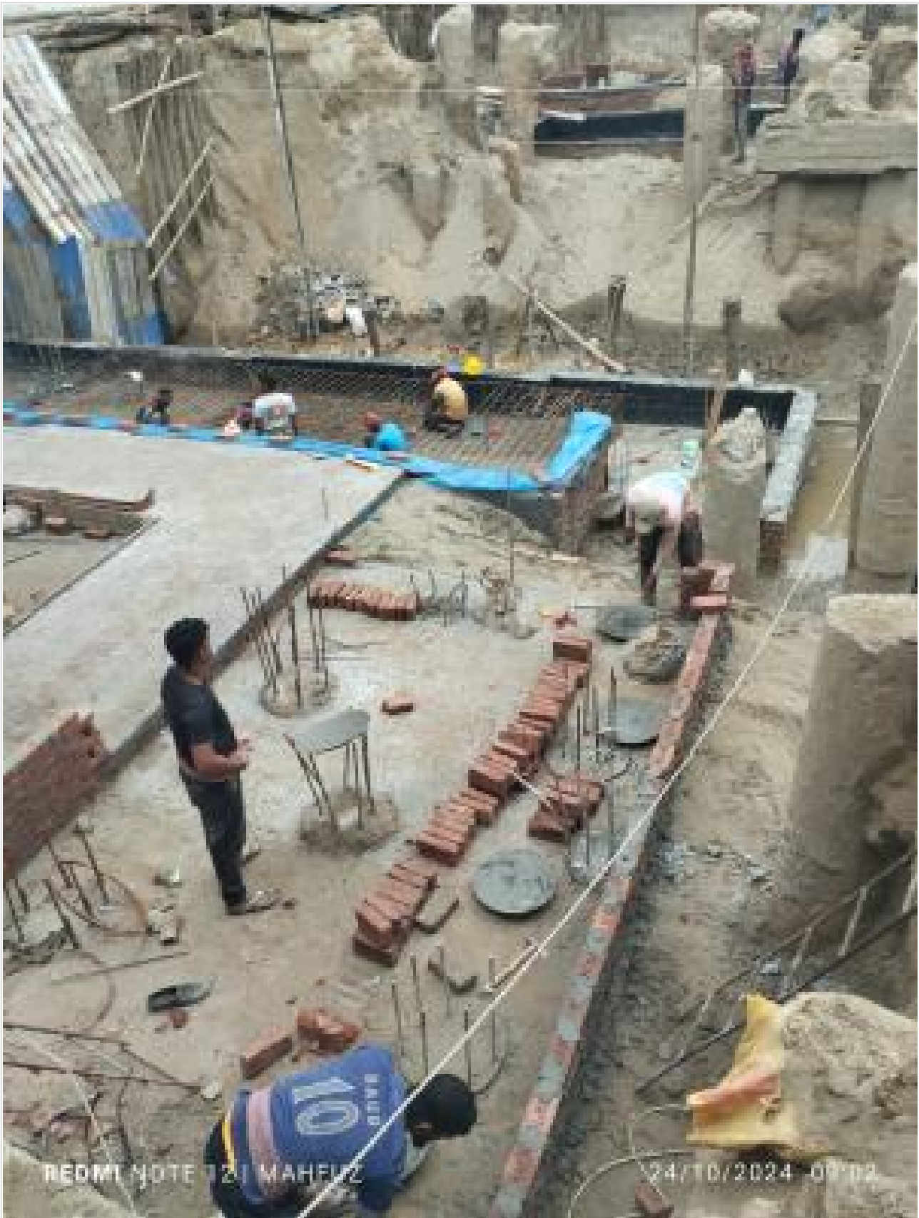
Tank base brick wall shuttering on 24-10-24
