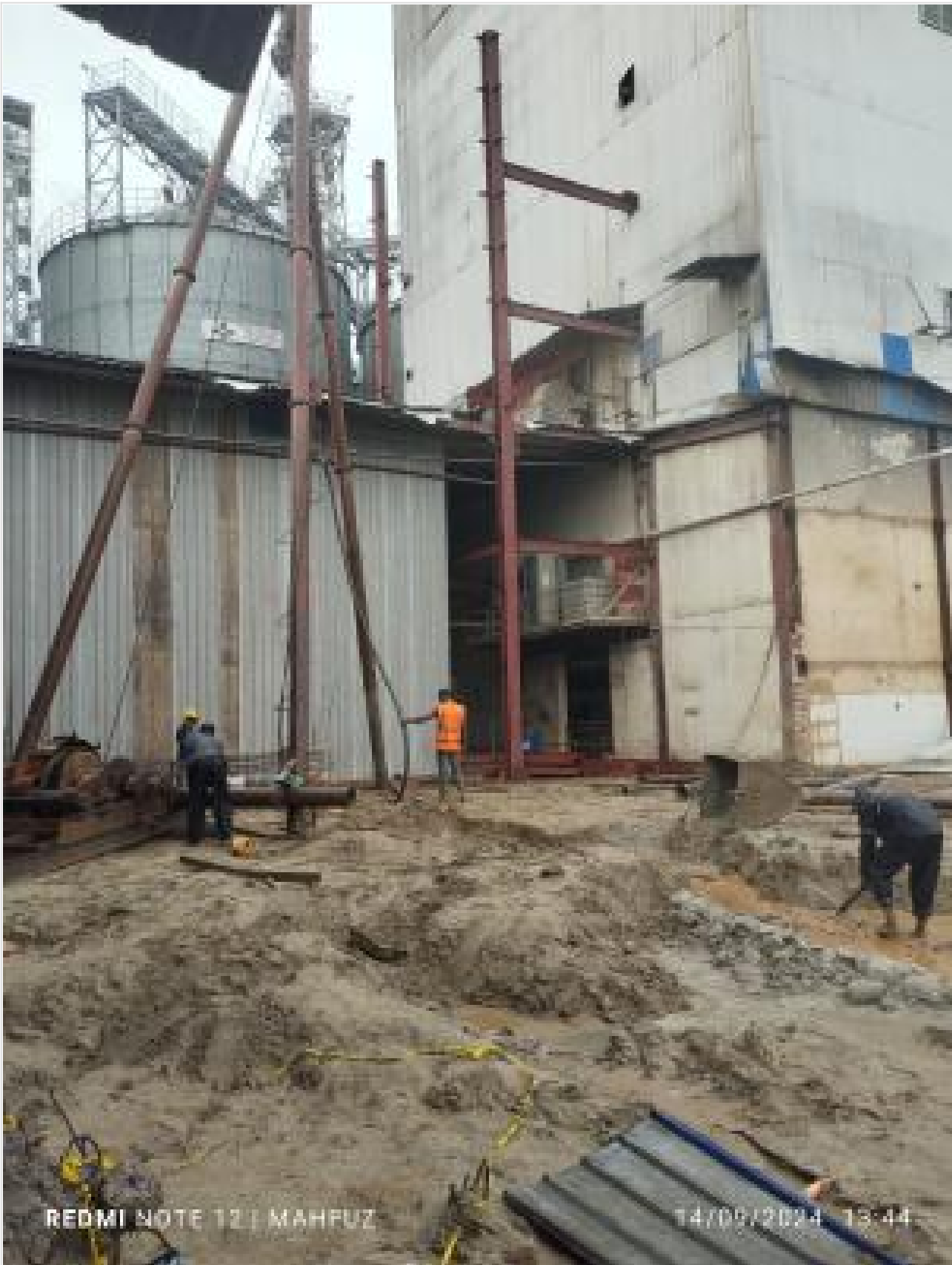
Pile boring on 14-09-24
