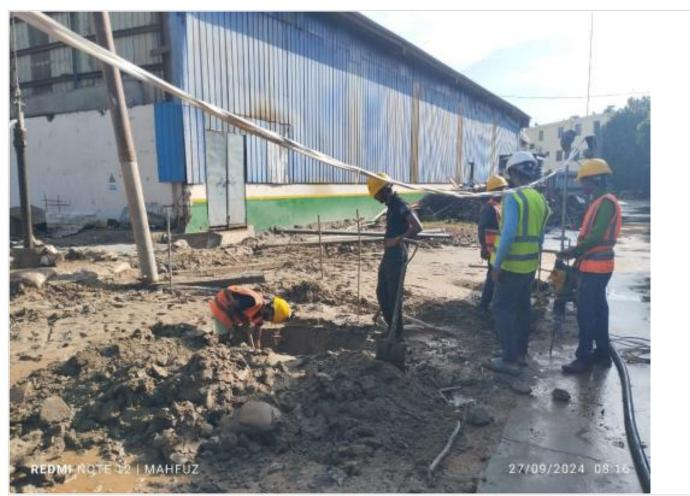
Excavating for pile boring obstacles on 27-09-24
