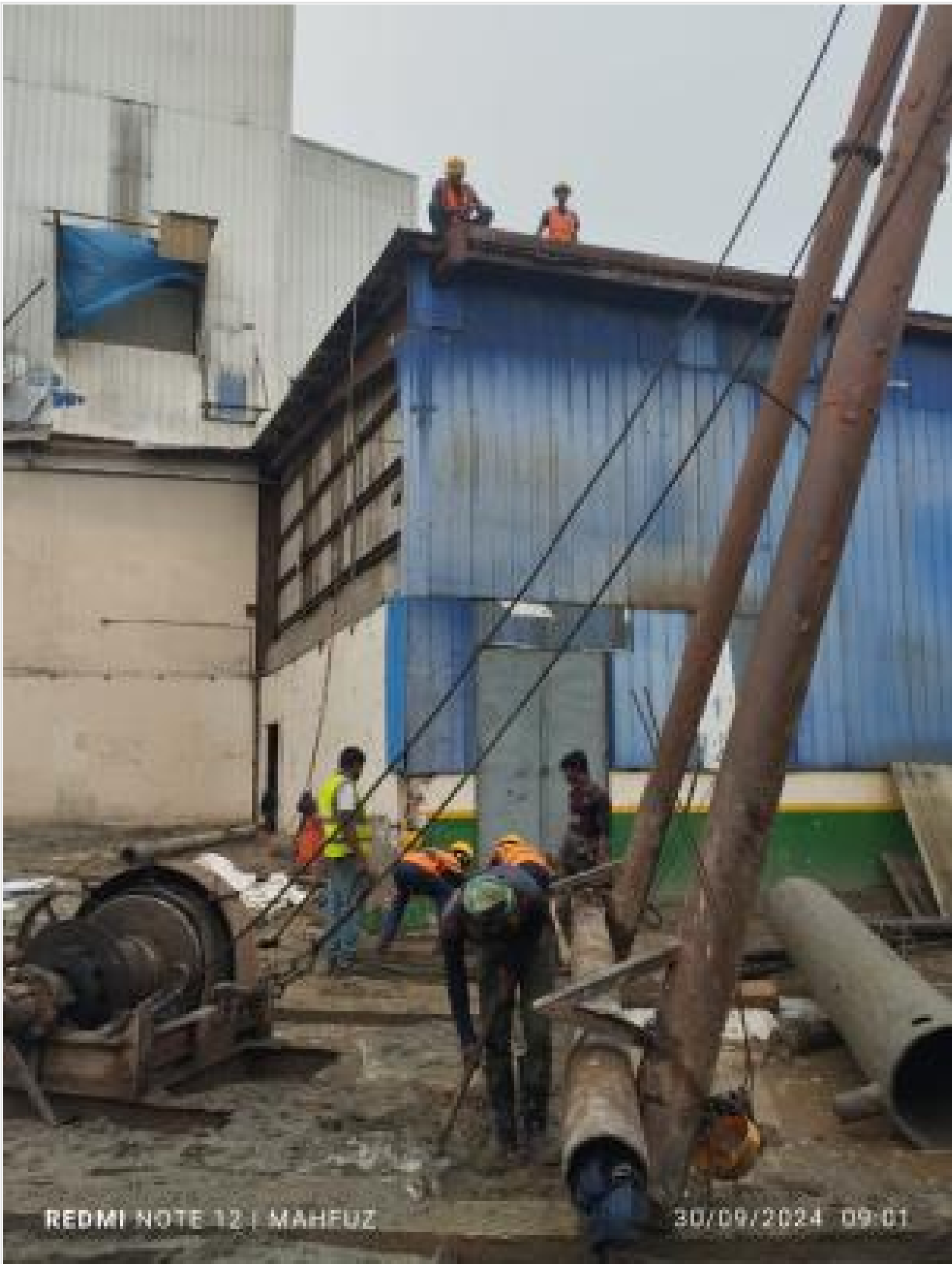
Piling rig shifting on 30-09-24
