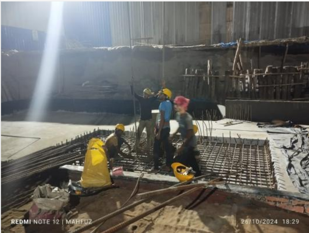
Pile cap re-bar work on 26-10-24
