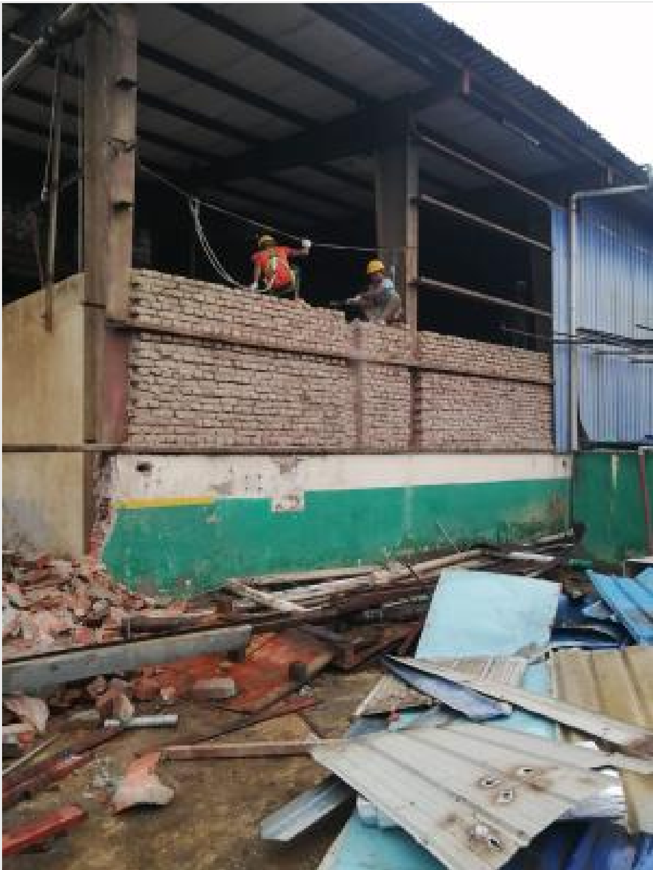
Brick wall dismatling on 03-09-24
