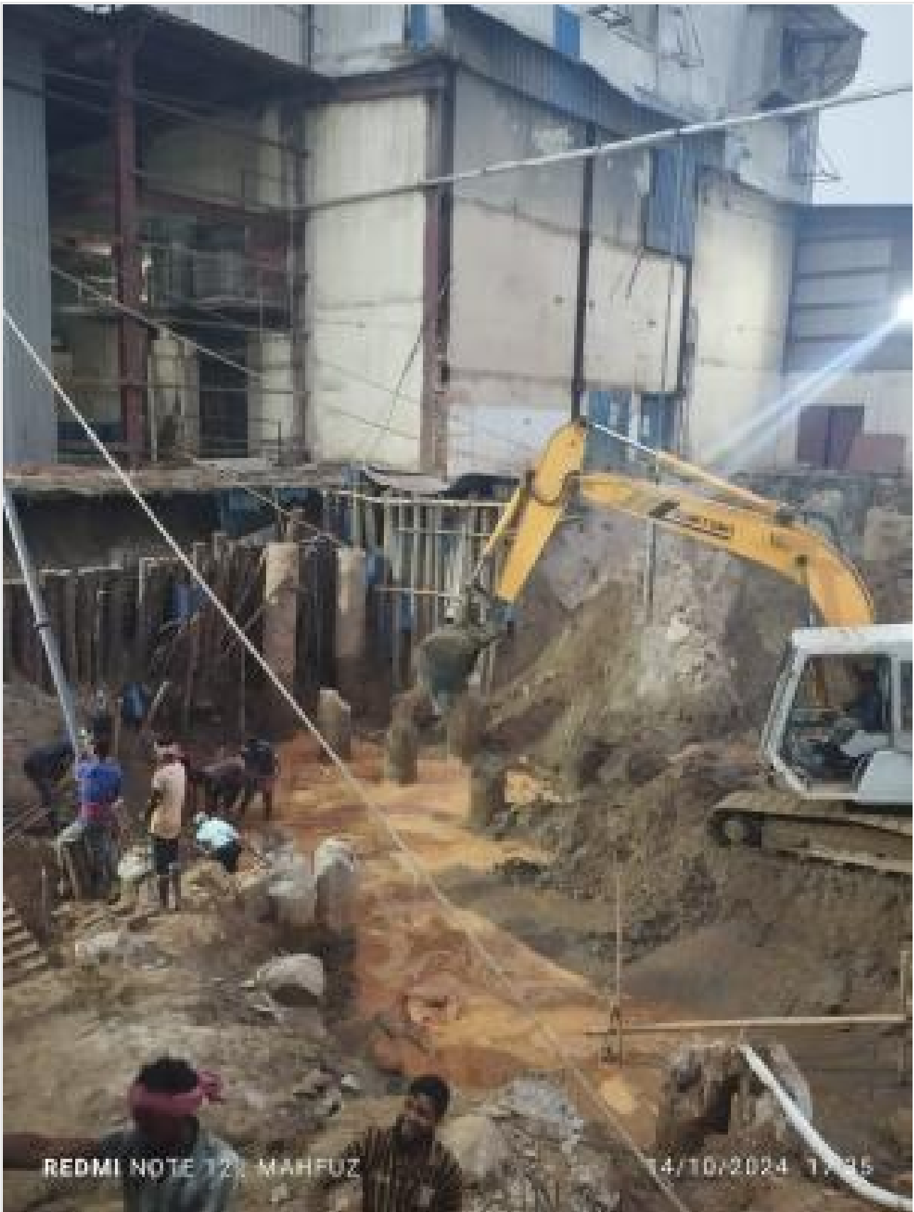
Earth excavation on 14-10-24
