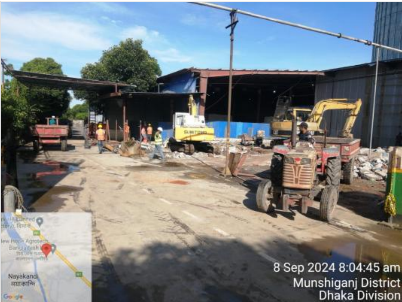
Floor,foundatn, road,tank cutting,removi on 08-09-24
