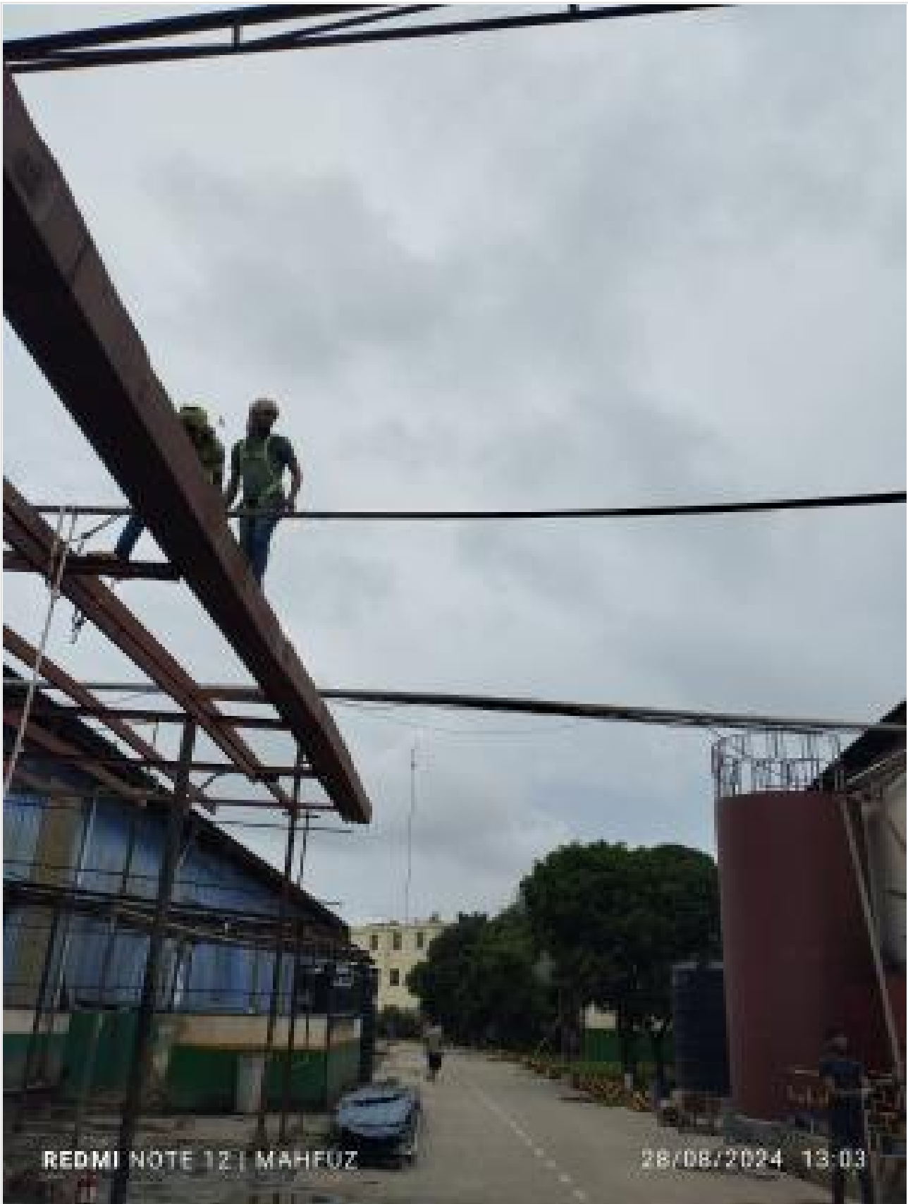
Sheet removing on 28-08-24
