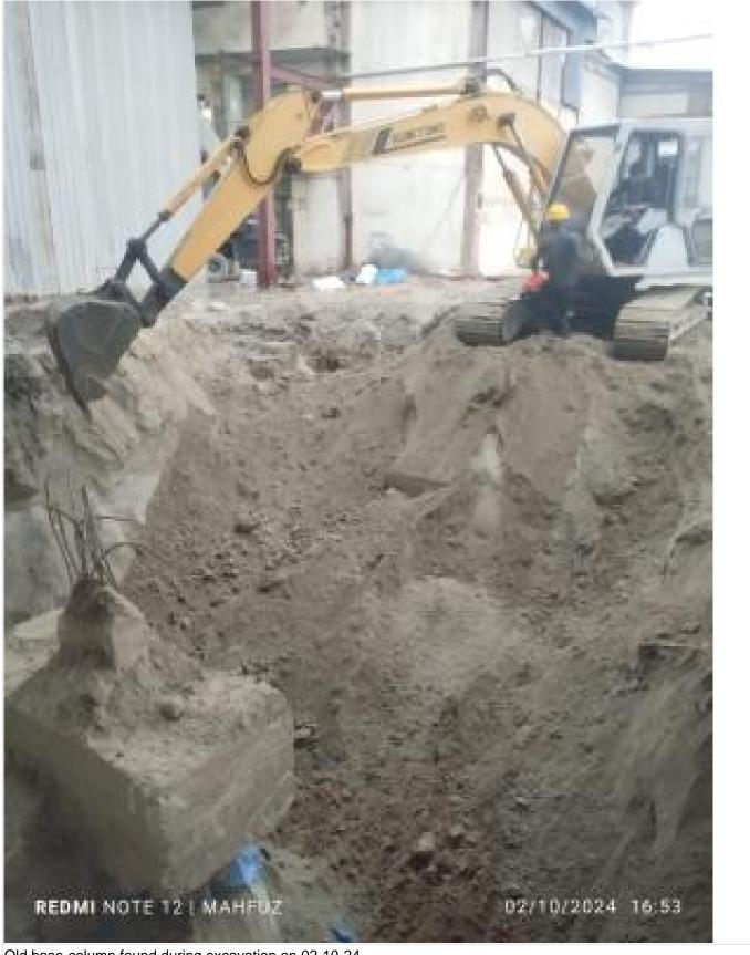
Old base-column found during excavation on 02-10-24 During excavating old foundation with column found In Grid-1 in between C and D
