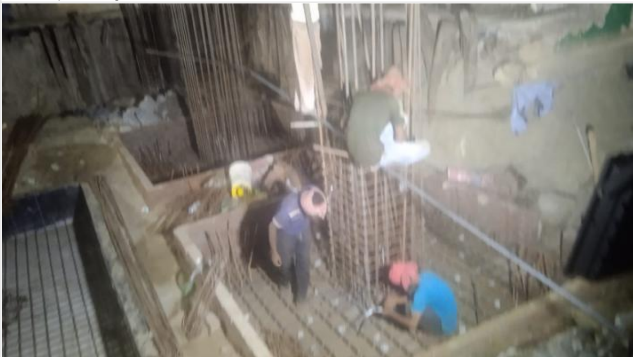
Raft re-bar work on 30-10-24
