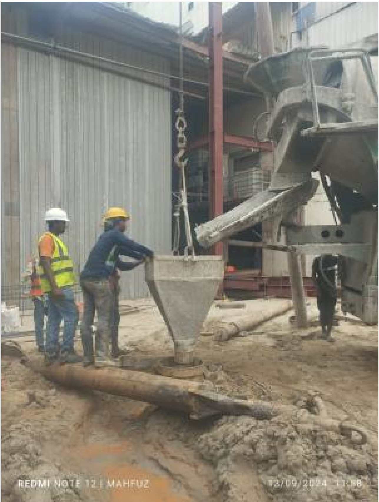
Pile concreting on 13-09-24
