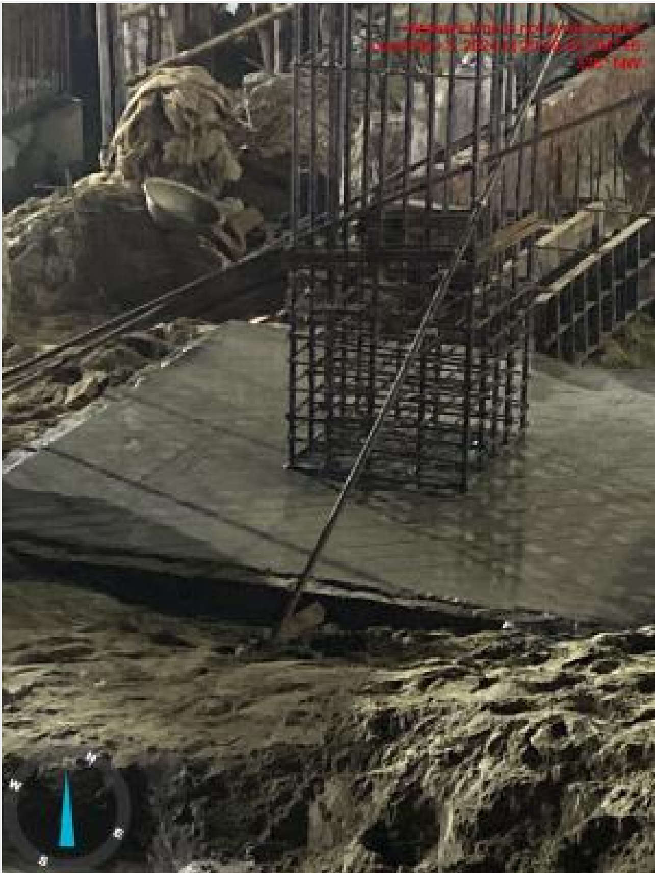
Pile cap concreting on 03-11-24
