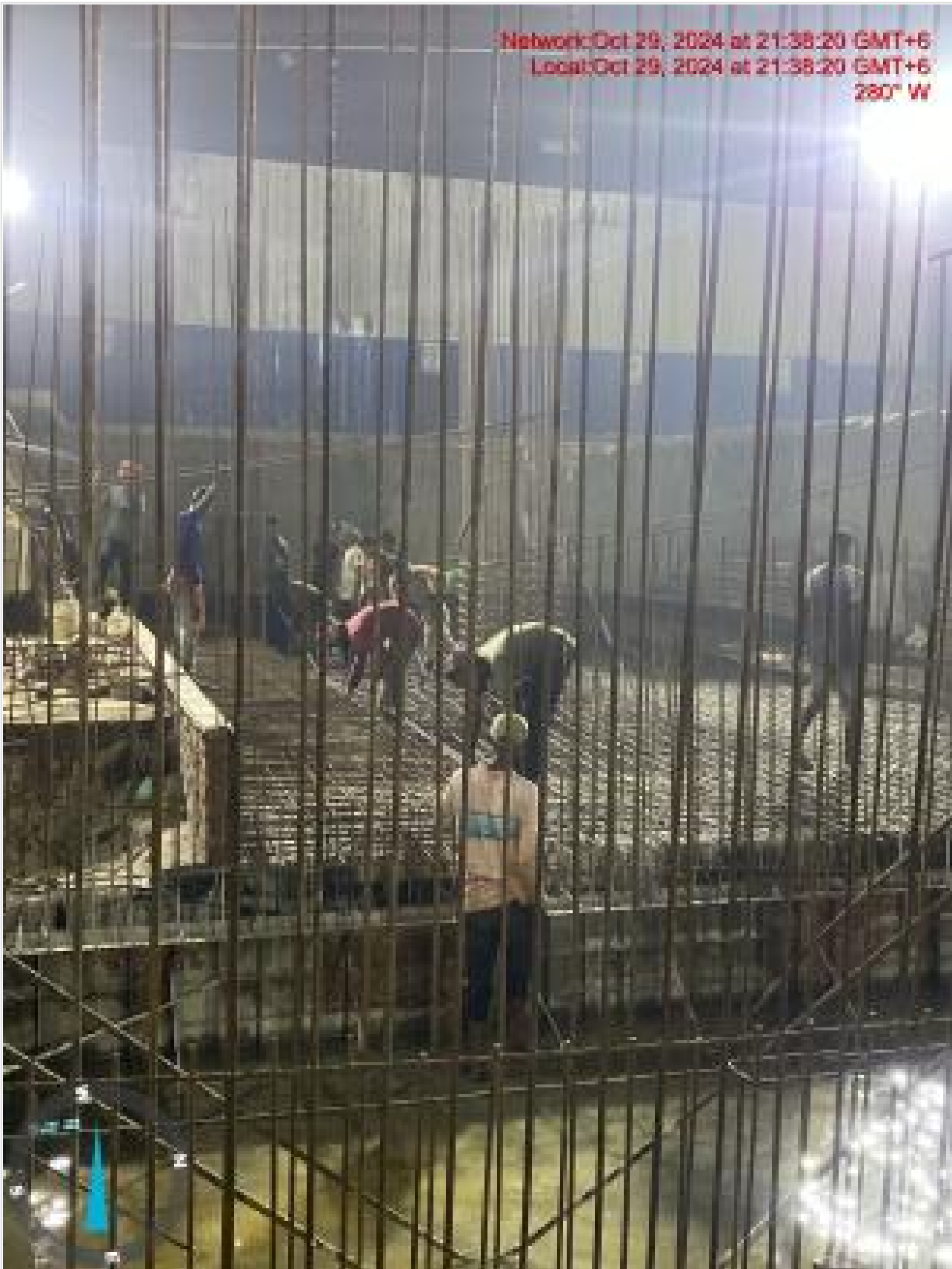
Raft re-bar work on 29-10-24
