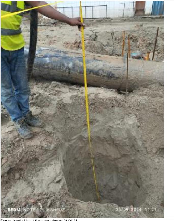
Due to electrical line 1.5 m excavation on 25-09-24 Due to live electric line Grid-3 Excavating all pile point upto 1.5 m
