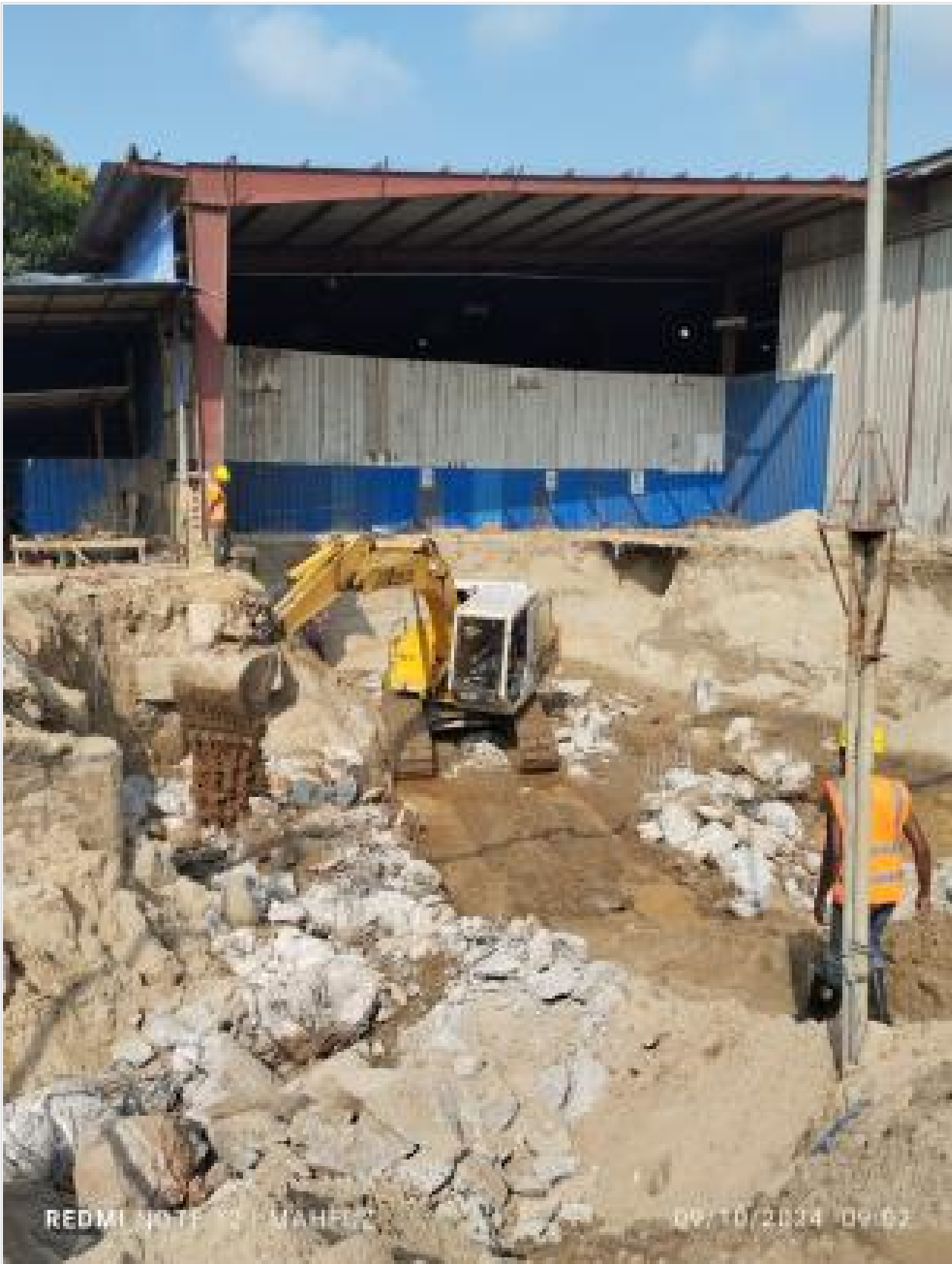
Earth excavation on 09-10-24
