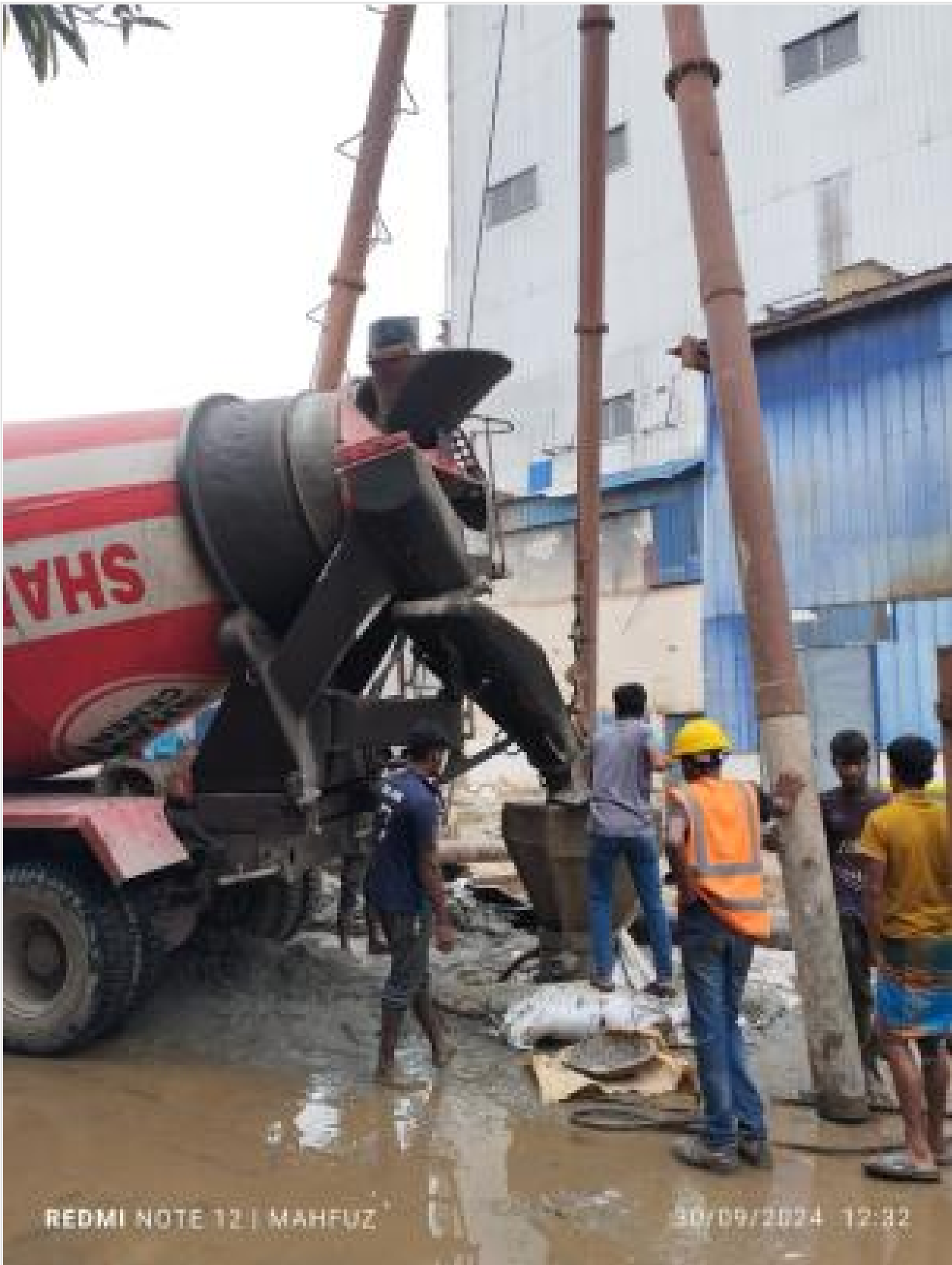
Pile concreting on 30-09-24
