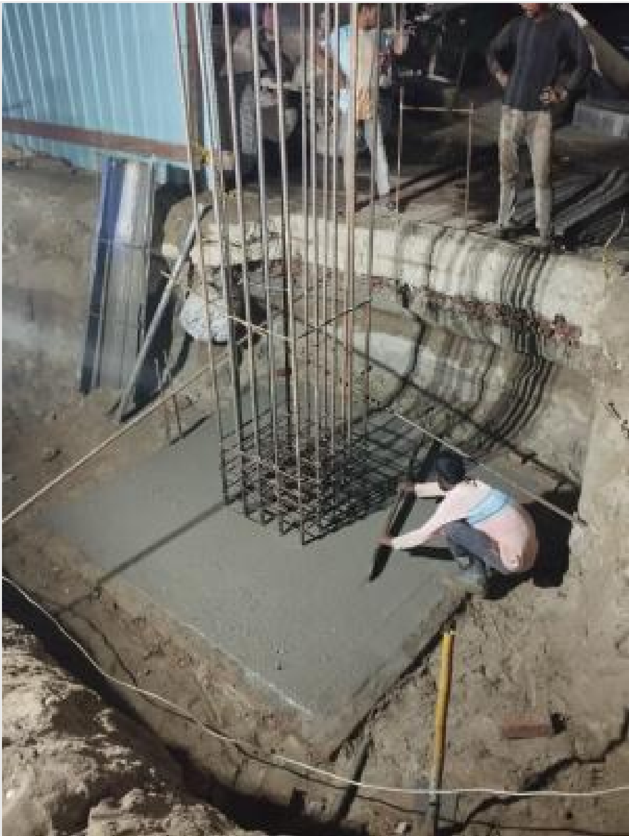
Pile cap concreting on 21-10-24
