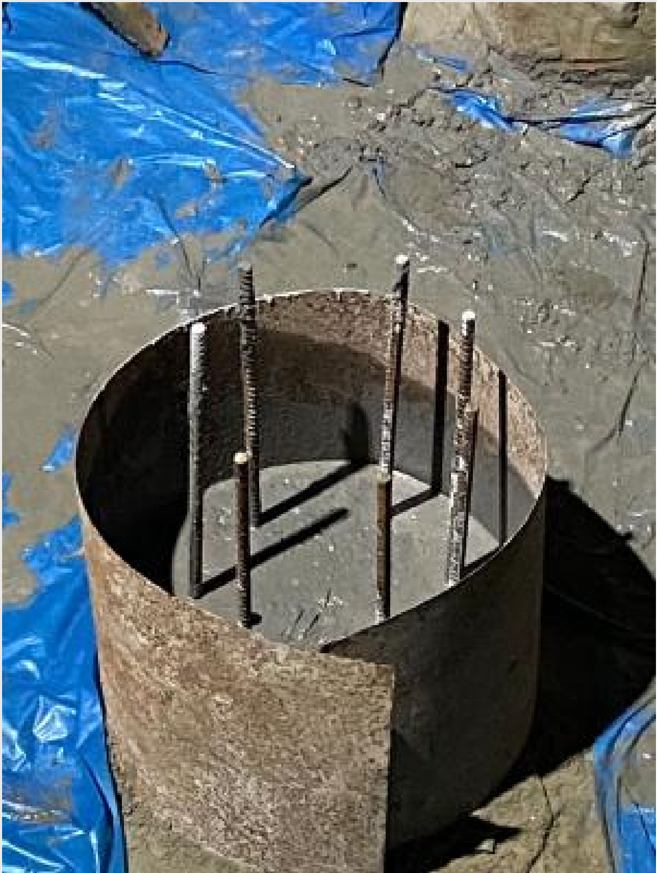
Pile Load Test-PDA-Pile Development on 10-10-24
