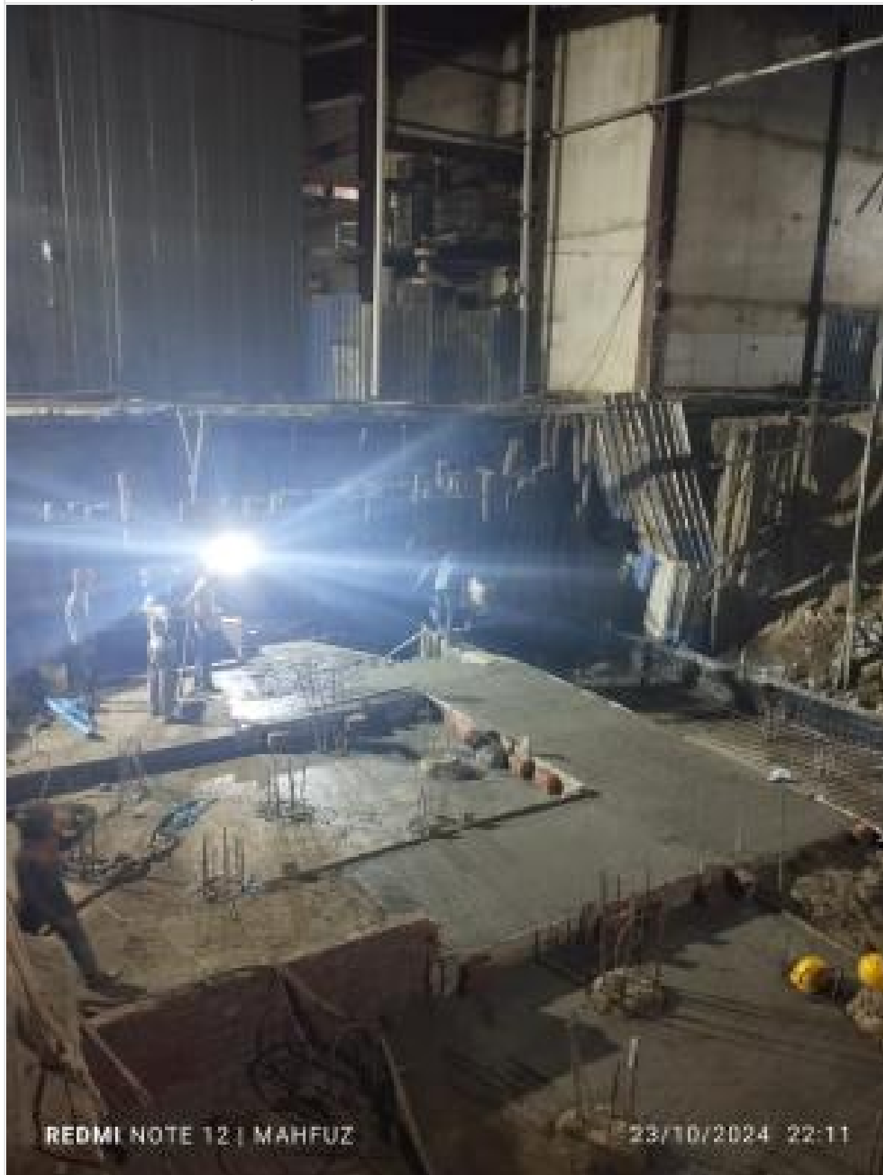
CC work on 23-10-24
