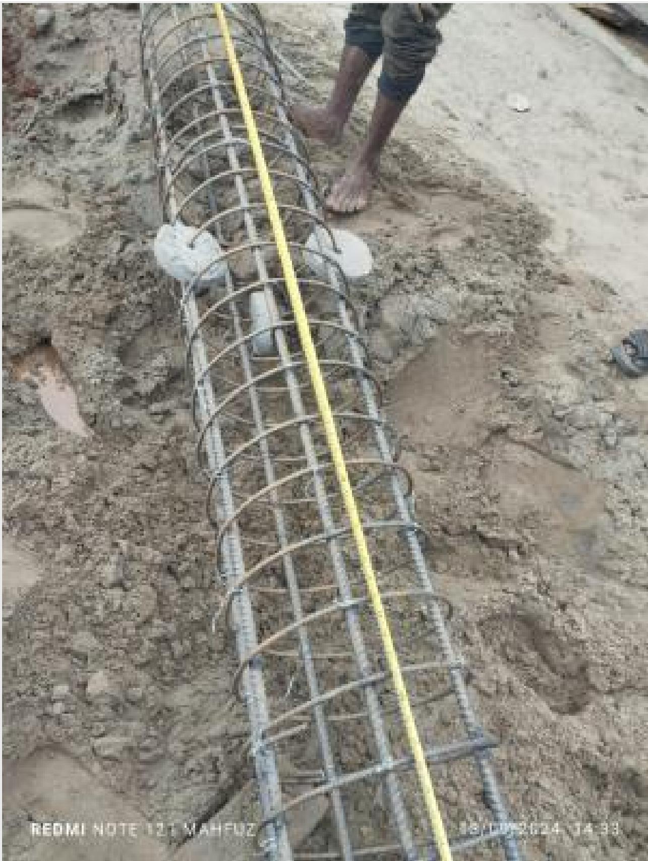
Pile cage length measuring on 13-09-24
