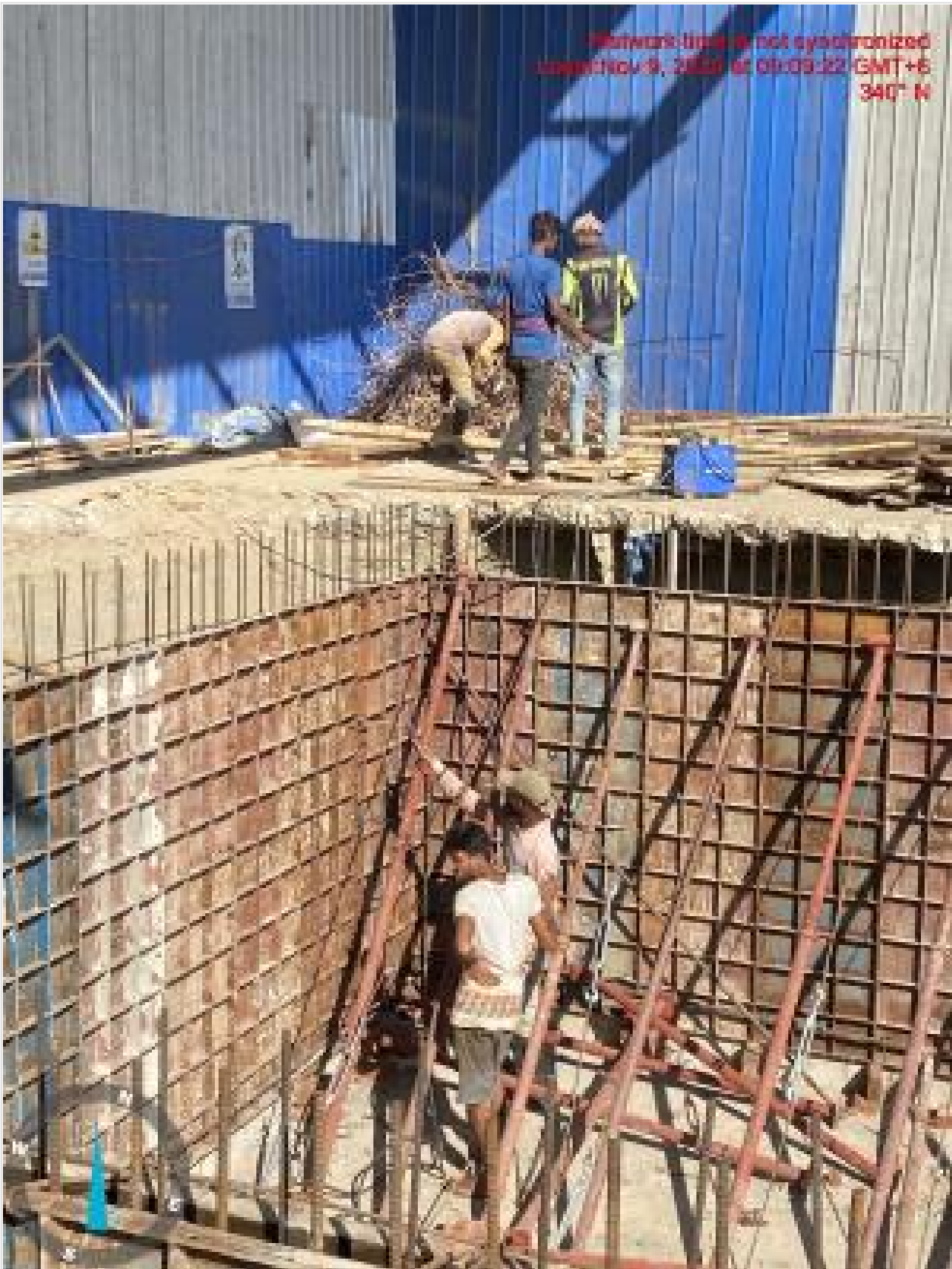
Wall shuttering on 09-11-24
