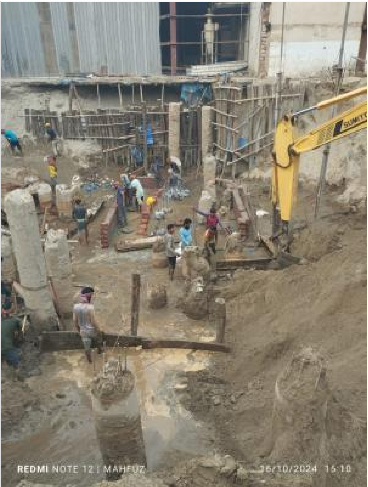
Excavation, brick-shuttering, steel shut on 16-10-24
