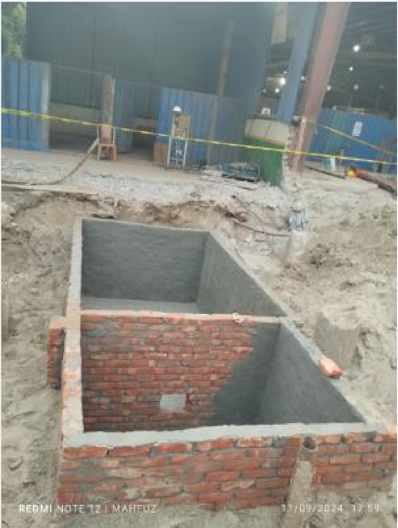
Pile mud tank complete on 11-09-24
