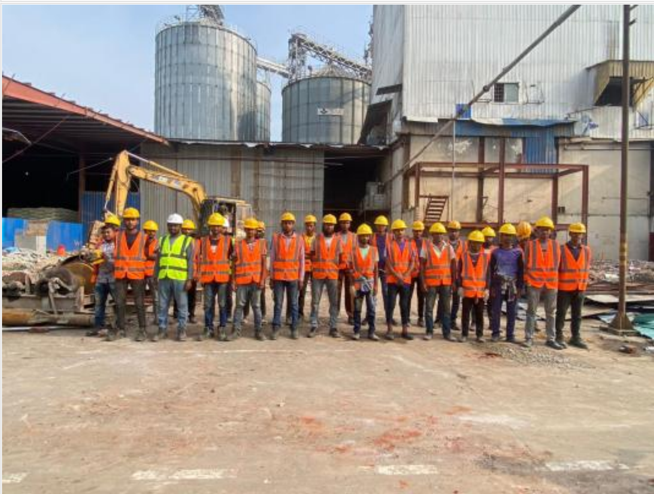
Steel Labour on 06-09-24
