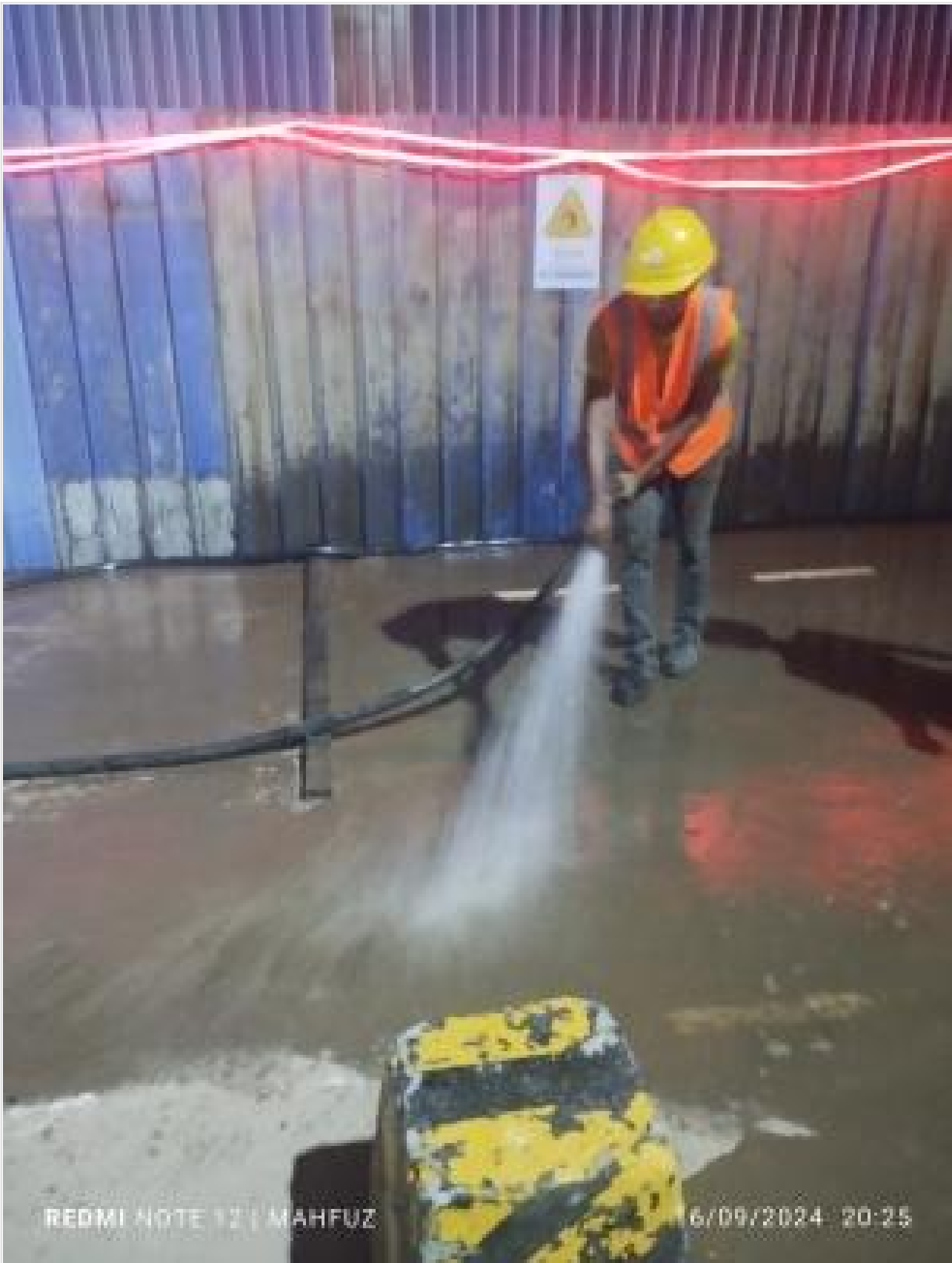
Road washing after pile finishing on 16-09-24
