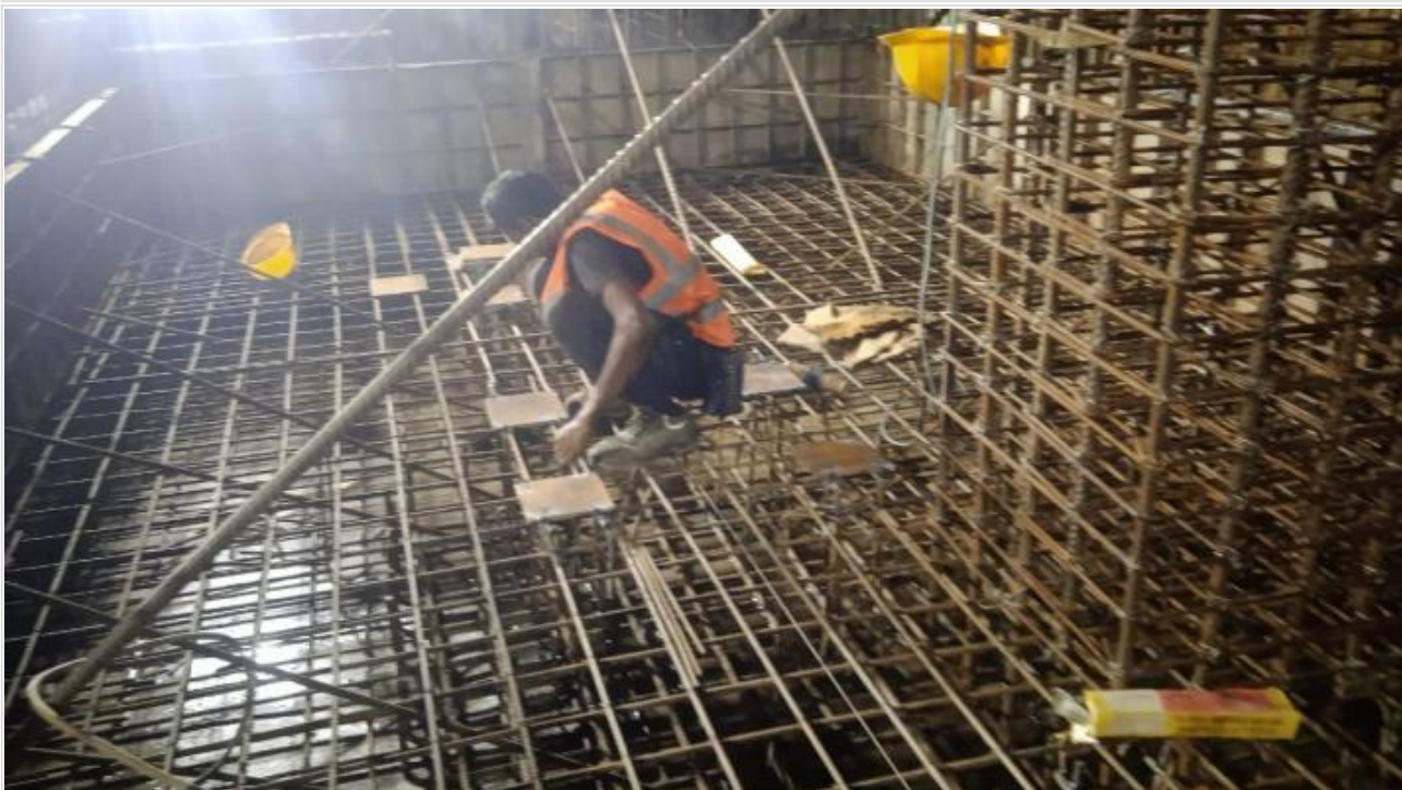
Pile cap re-bar work on 27-10-24
