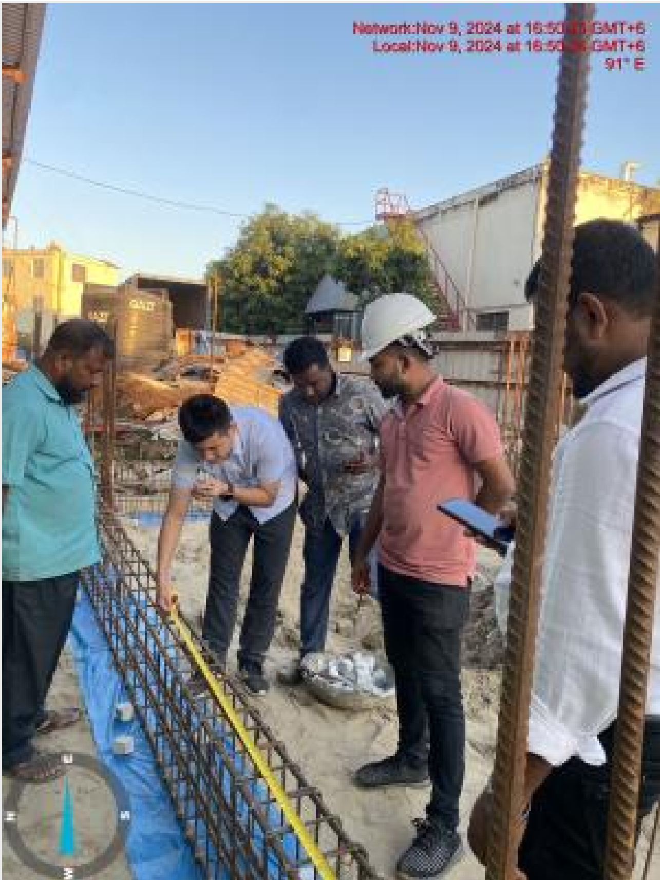
Foundation beam rebar inspection on 09-11-24
