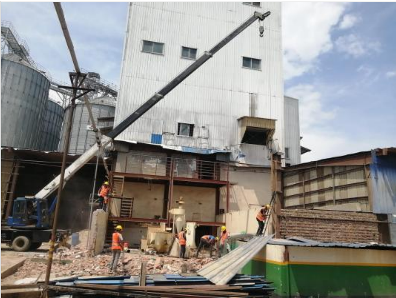
Material shifting by crane on 05-09-24
