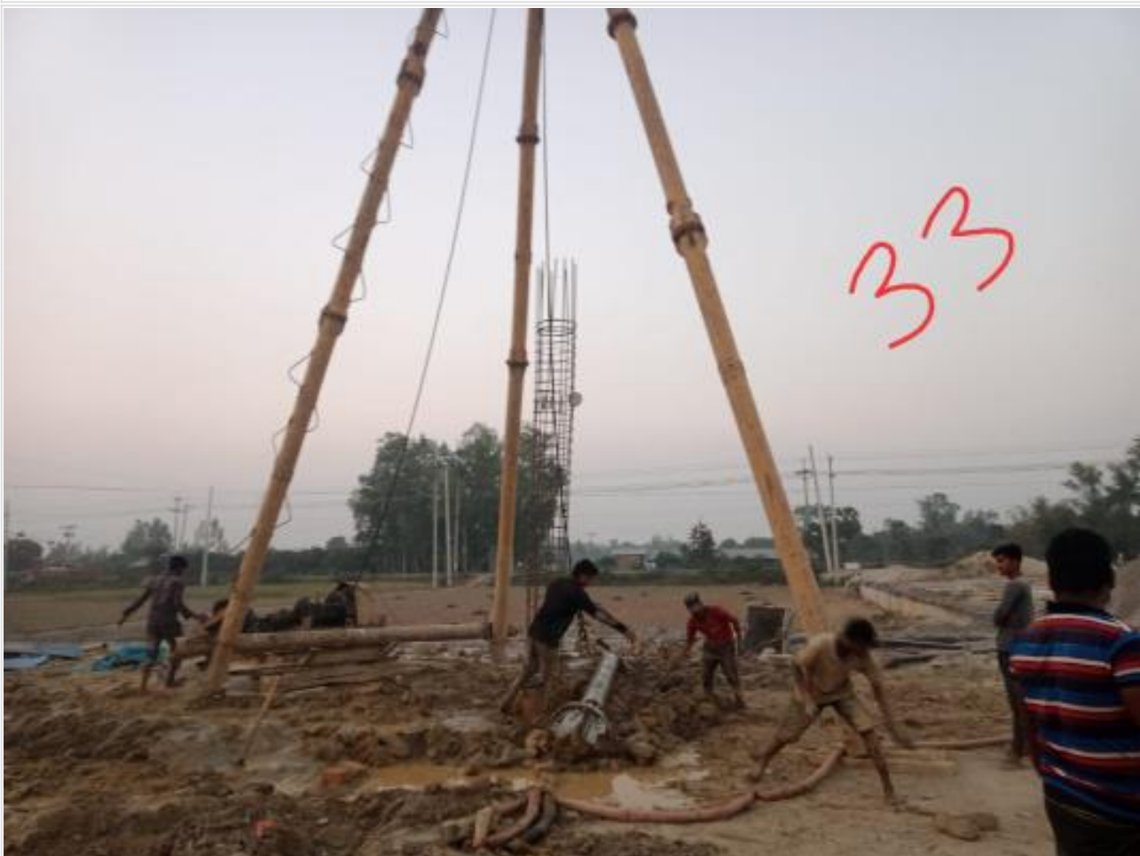
Com. Bldg. 33 pile boring on 27-02-23
