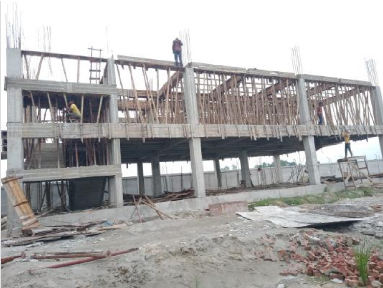
Dorm. Bldg. 2nd floor Shuttering work on 04-09-23
