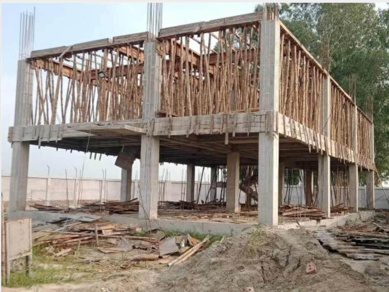
Dorm. Bldg. 2nd floor shuttering work on 03-09-23
