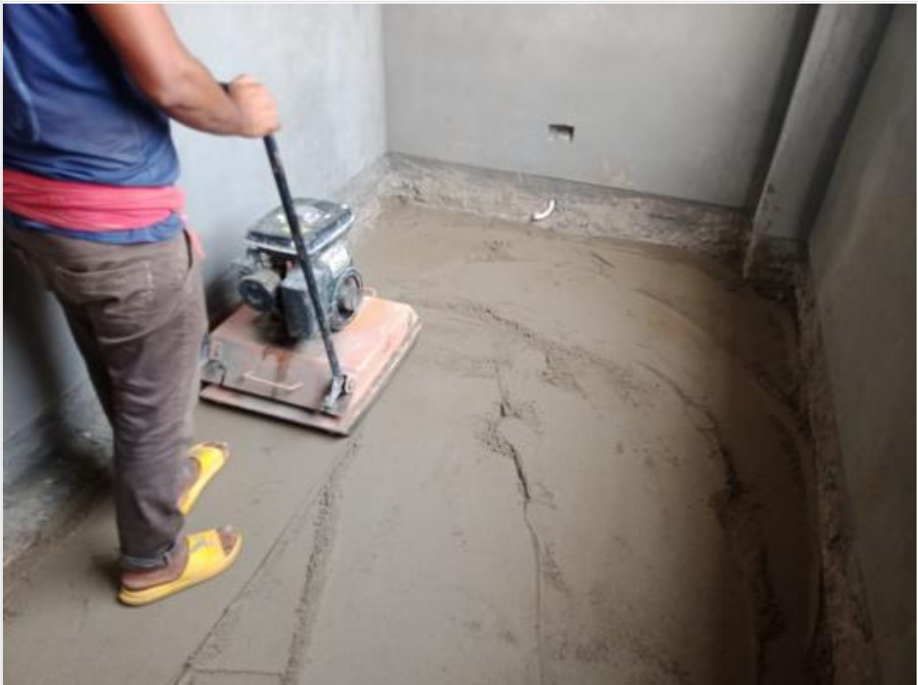
Dorm. Bldg. GF sand khoa cushion on 09-11-23
