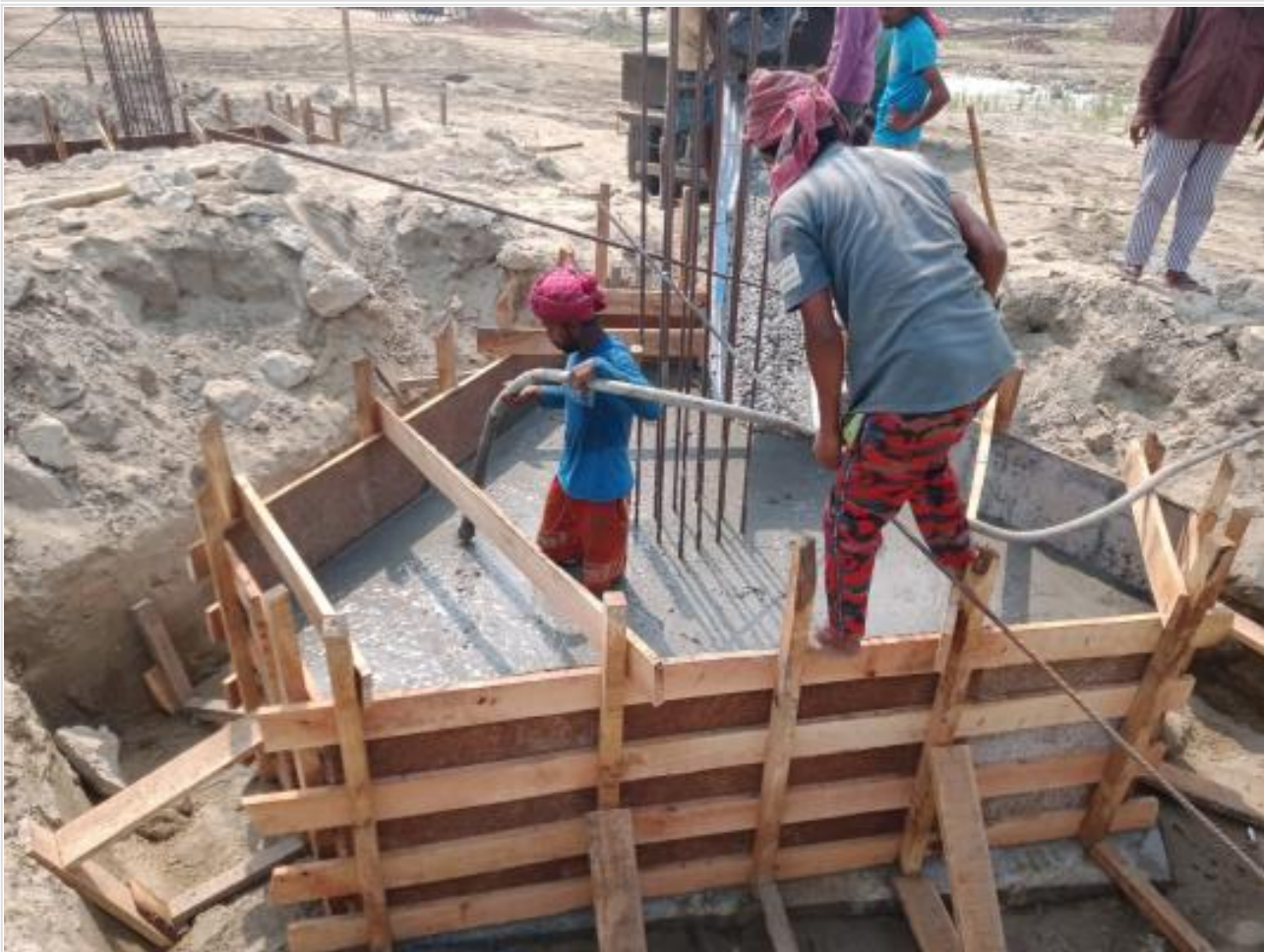
Comp. Bldg. Pile cap casting on 16-04-23
