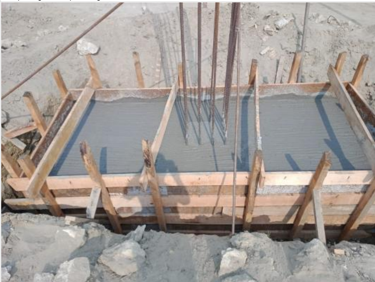
Pile Cap concreting. on 16-04-23
