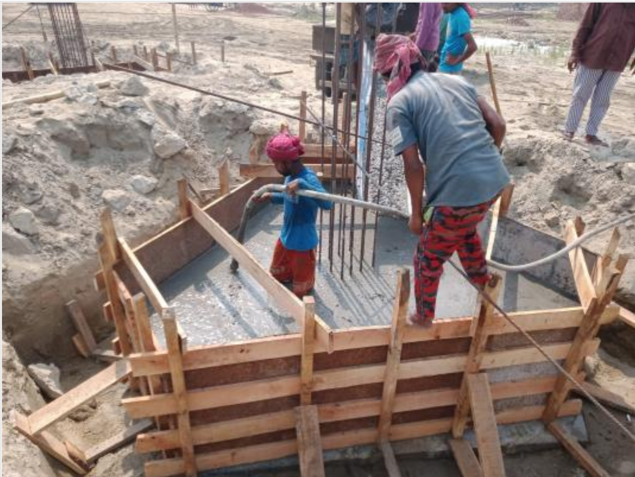
Comp. Bldg. Pile cap casting on 16-04-23
