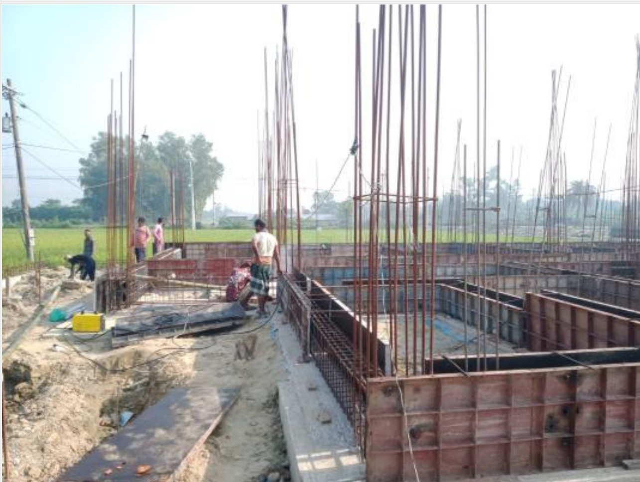
Comp. Bldg. GB Shuttering work on 08-05-23
