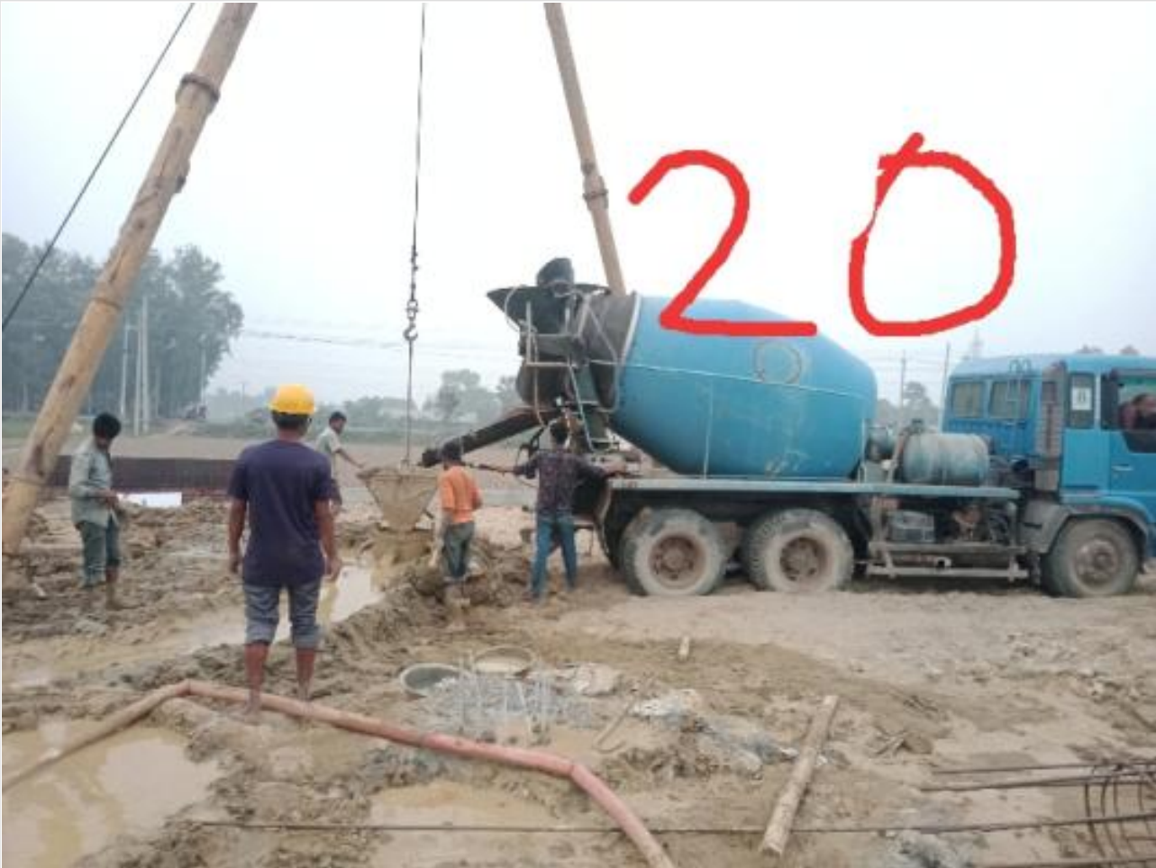
Ready mix concreting of pilewort on 22-02-23
