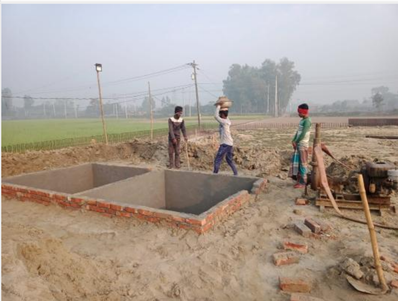
Mud Tank-1 Completed on 08-02-23
