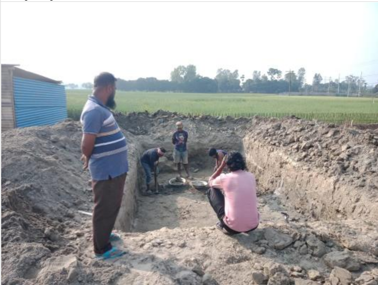
Excavation for Pile Mud Tank on 03-02-23
