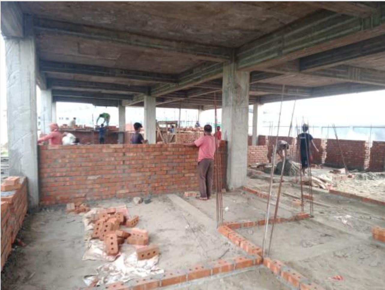
Dorm.Bldg brick work on 23-09-23
