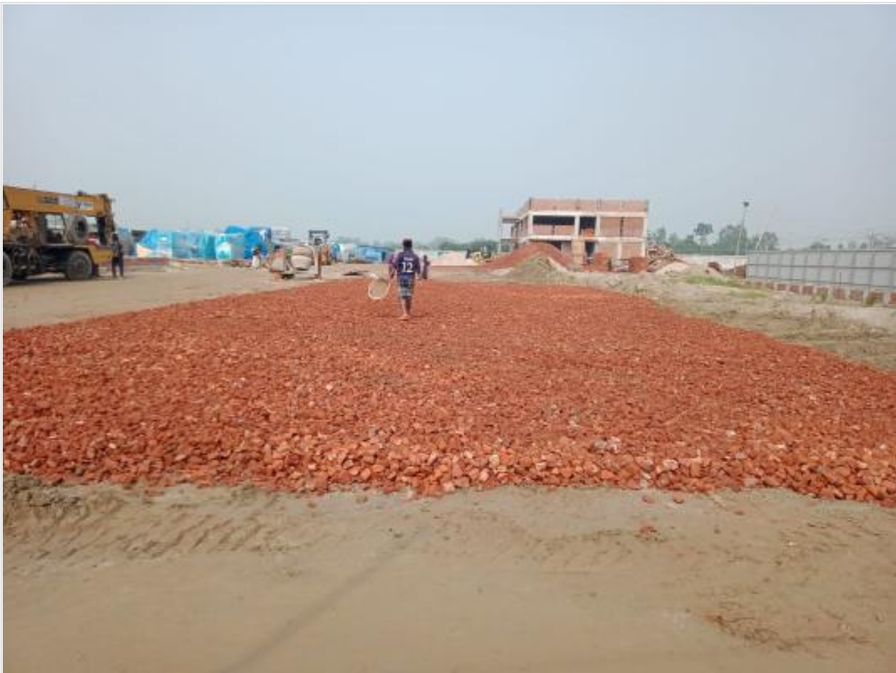
Road Sub-base work on 01-09-23
