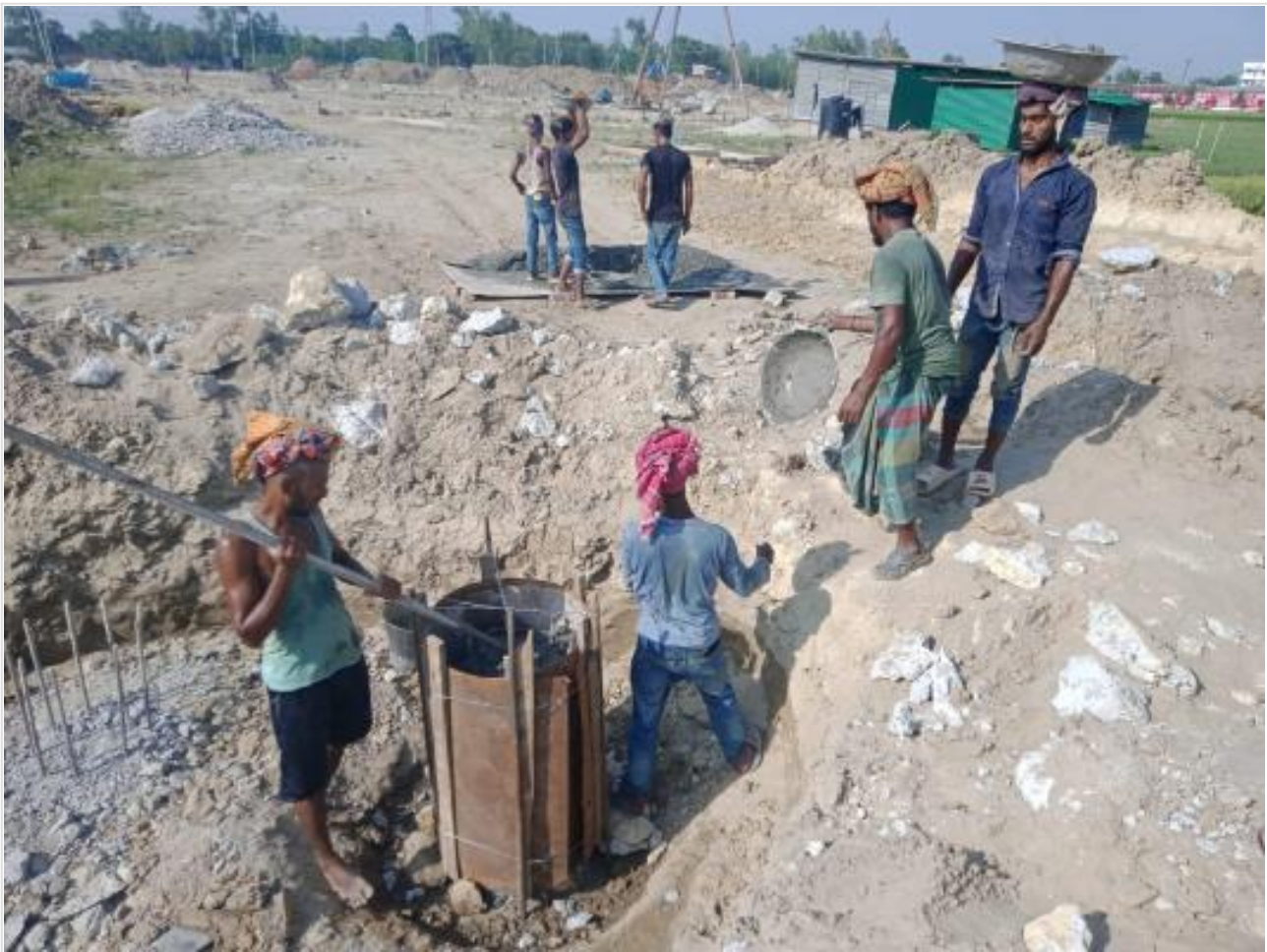
Pile head finishing for test on 09-05-23
