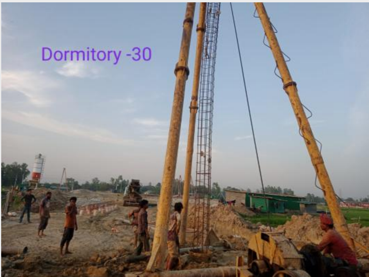
Pile head finishing for test on 07-04-23
