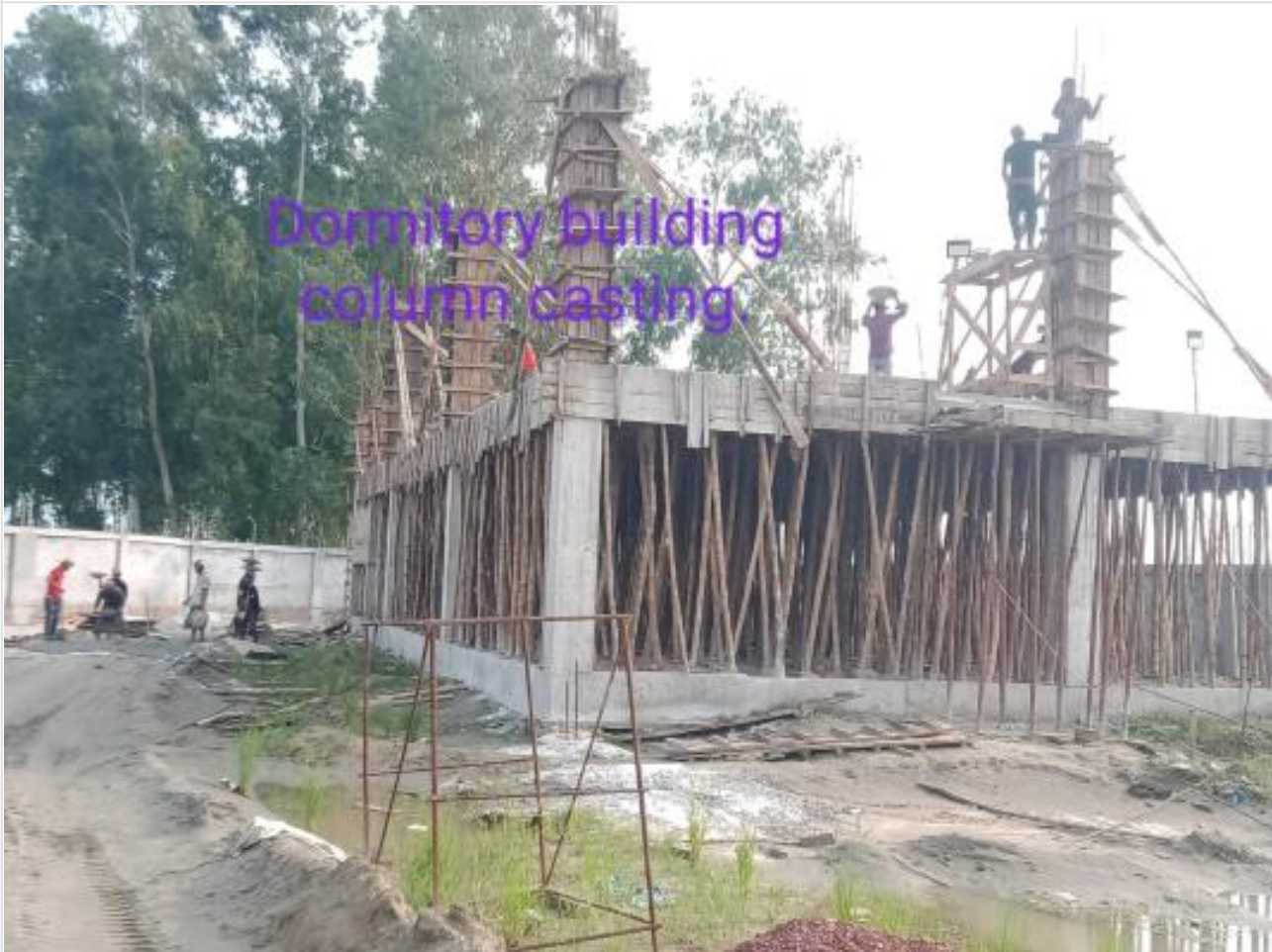
Dormitory Column Concreting on 23-08-23
