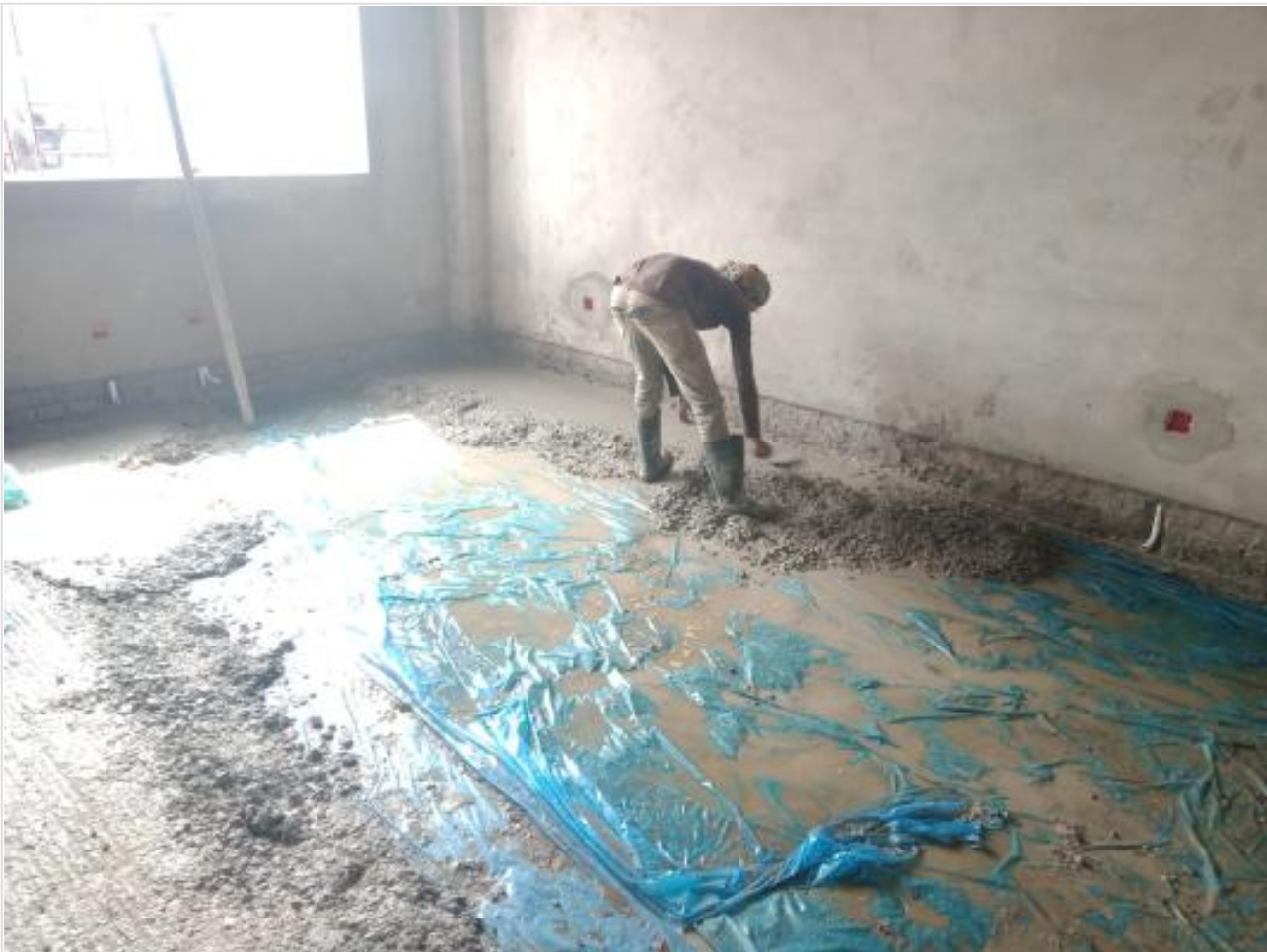
Comp. Bldg. GF casting on 09-10-23
