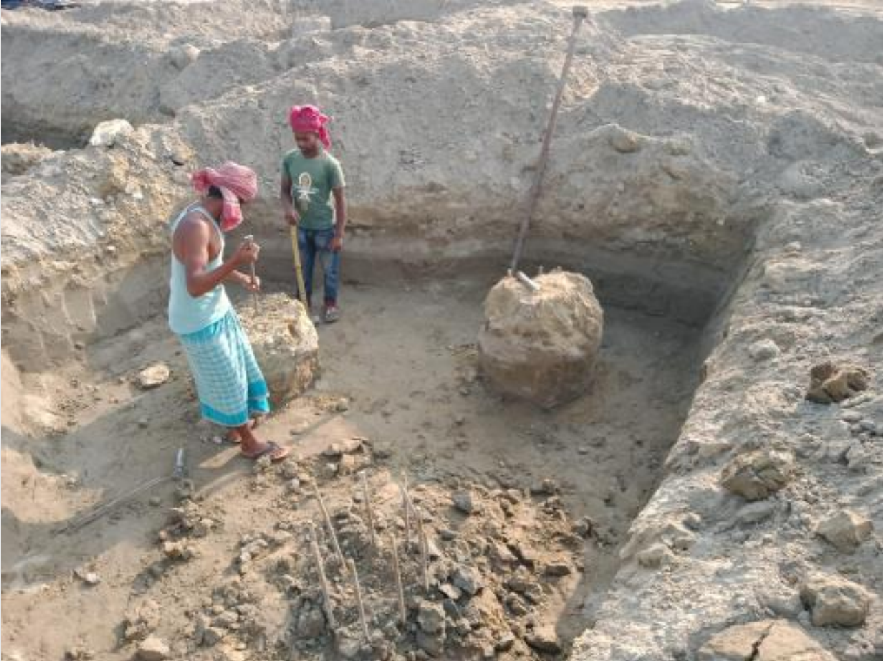
Pile cap earth cutting on 27-03-23
