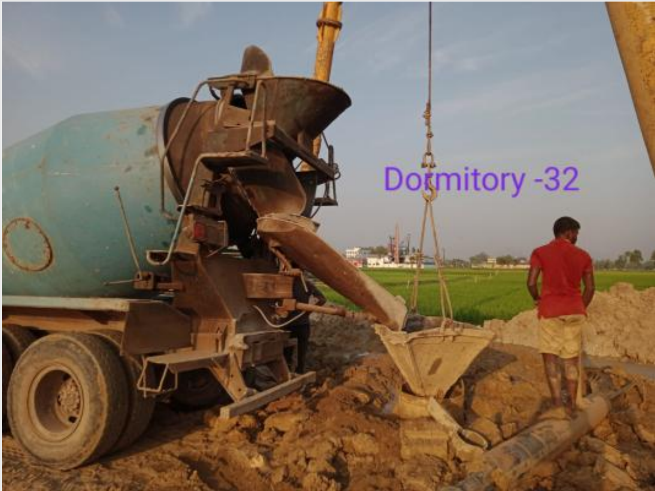
Dorm. Bldg. 32nd pile concreting on 09-04-23
