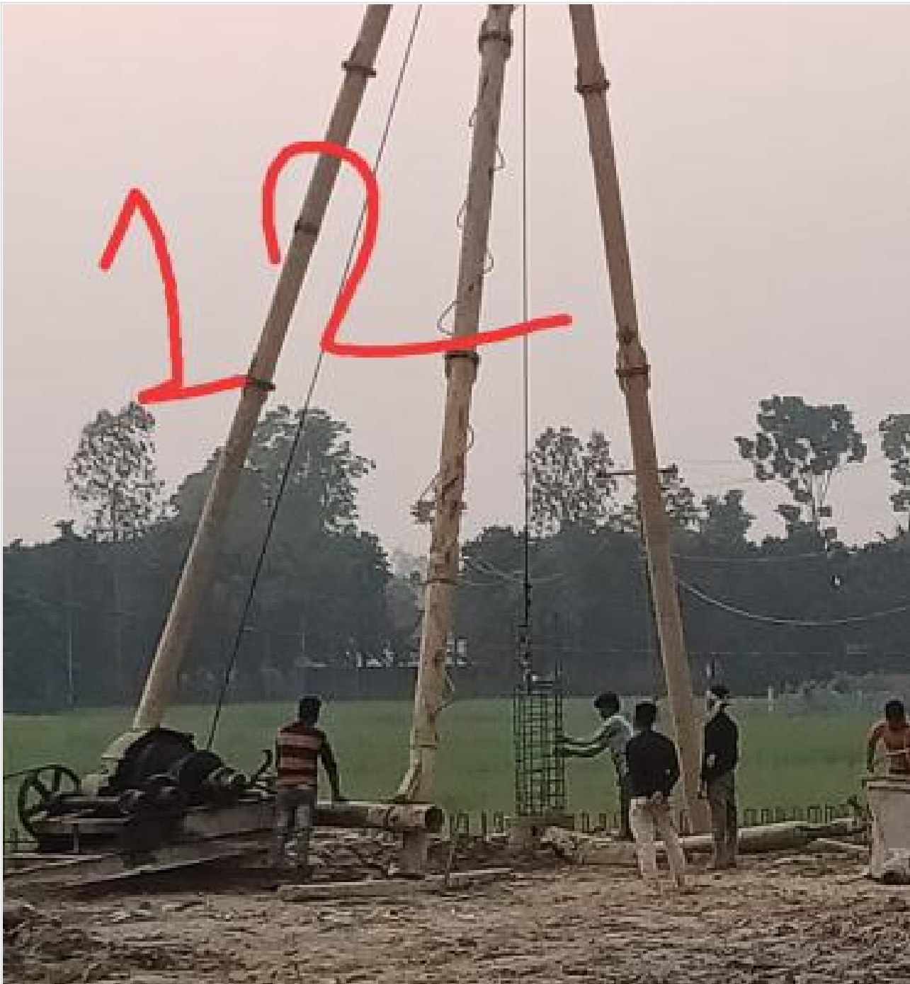
Com. Bldg. 12th pile boring on 17-02-23
