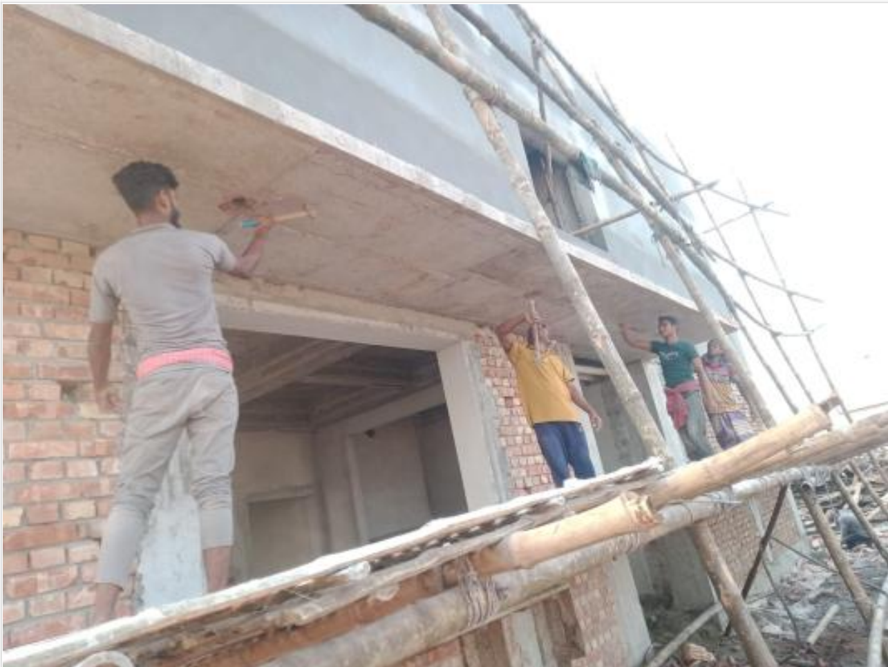
Comp. Bldg. Outside plaster work on 13-10-23
