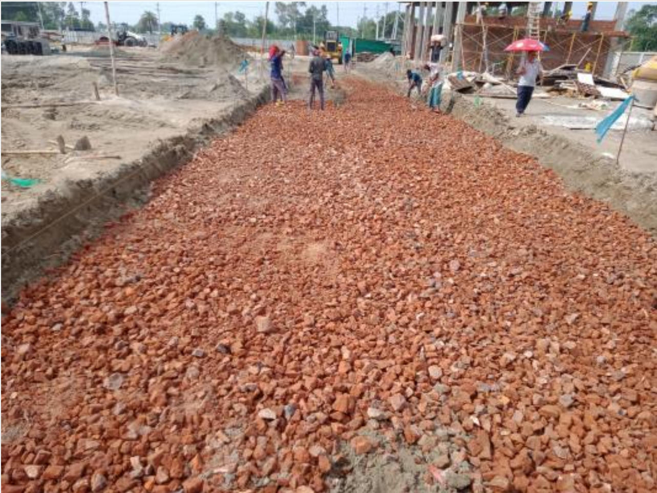
Road-Sub-base work on 21-08-23
