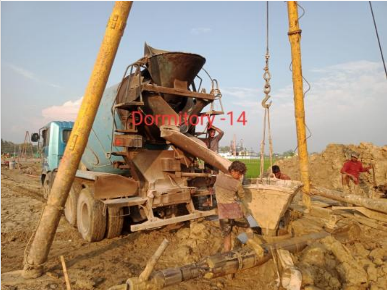
Ready mix concreting of pile on 01-04-23
