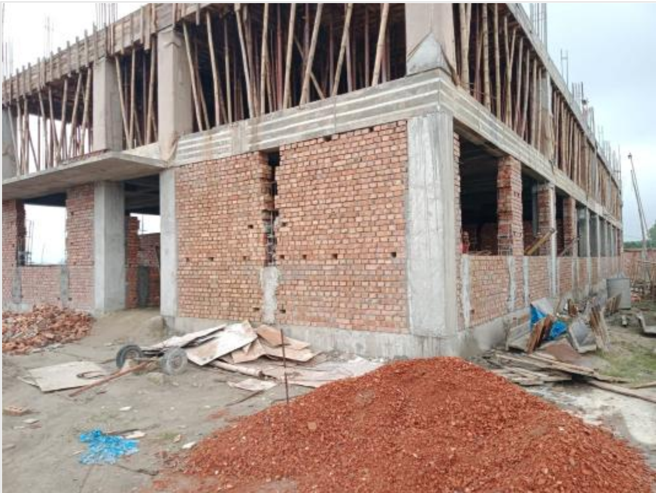
Comp.Bldg GF Brick work on 06-08-23
