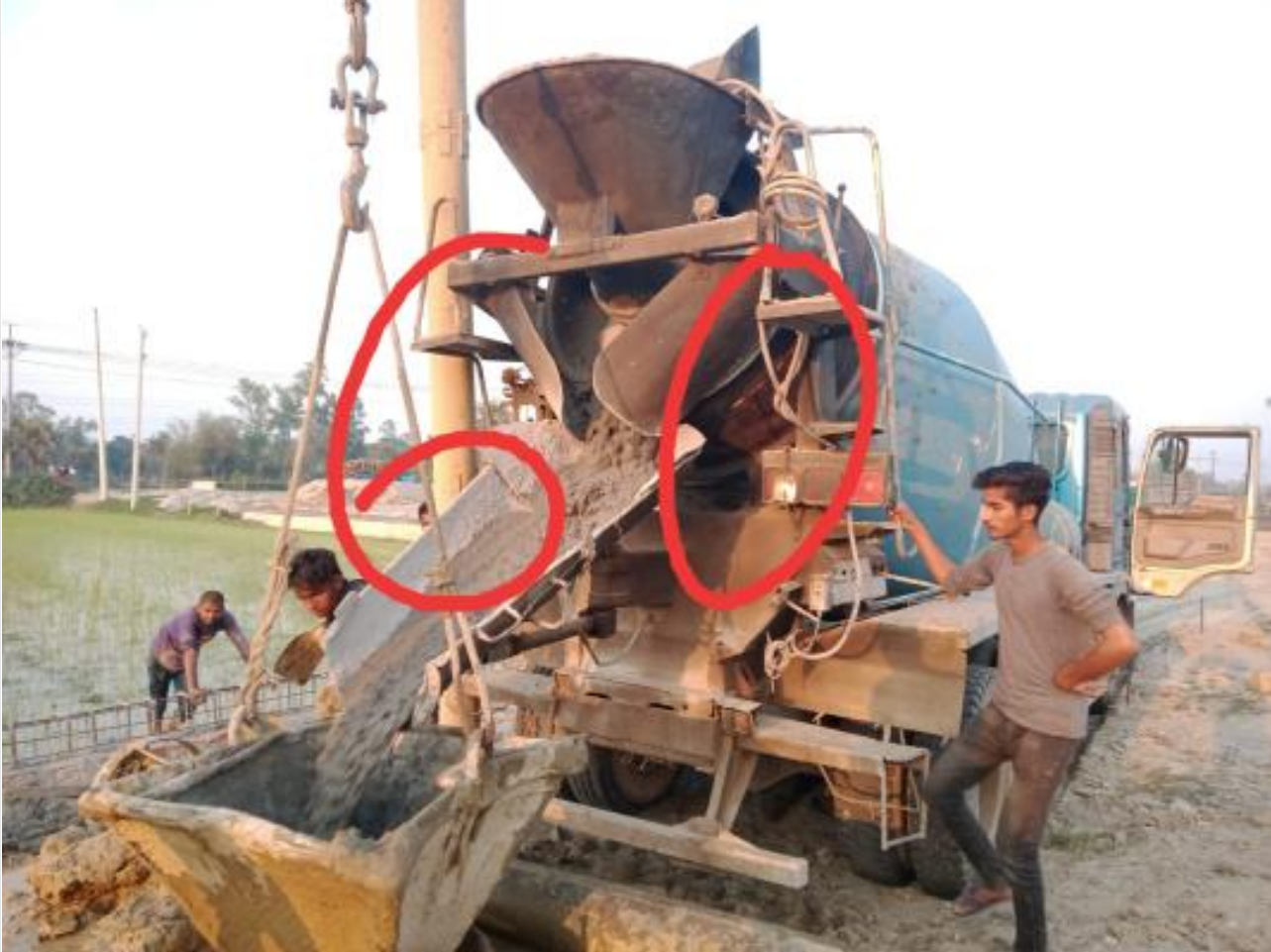
Ready mix concreting of pile on 13-03-23
