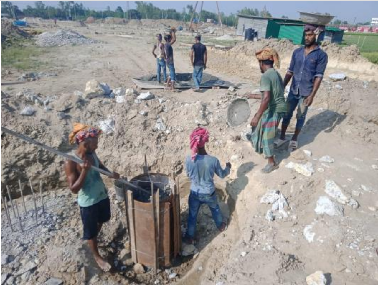
Pile head finishing for test on 09-05-23
