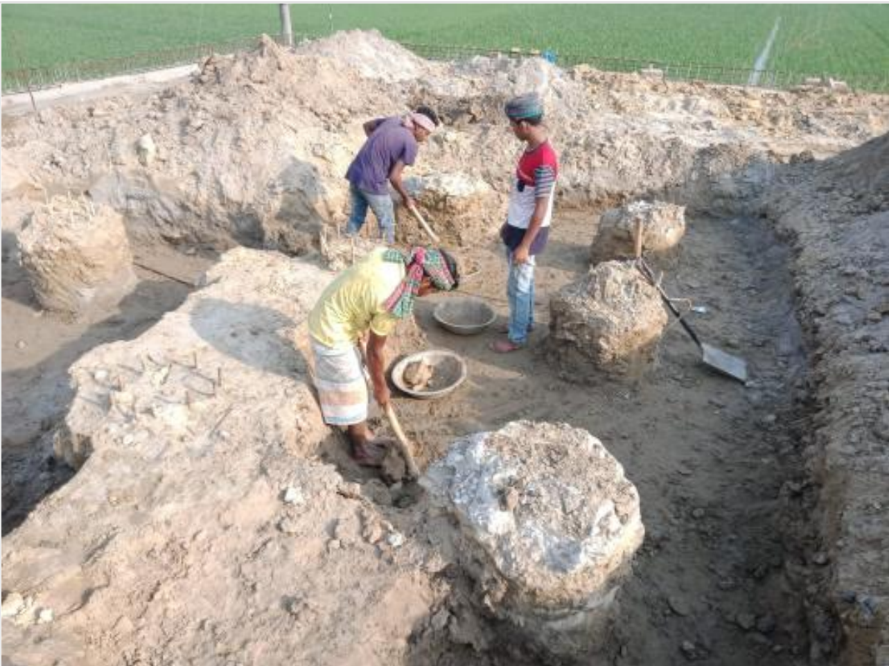
Pile cap earth cutting on 27-03-23
