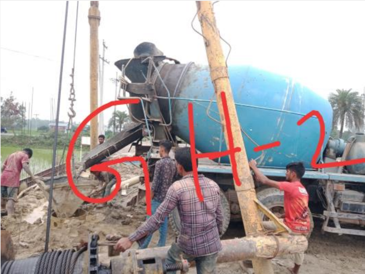
Guard House pile concreting by RMC on 19-03-23
