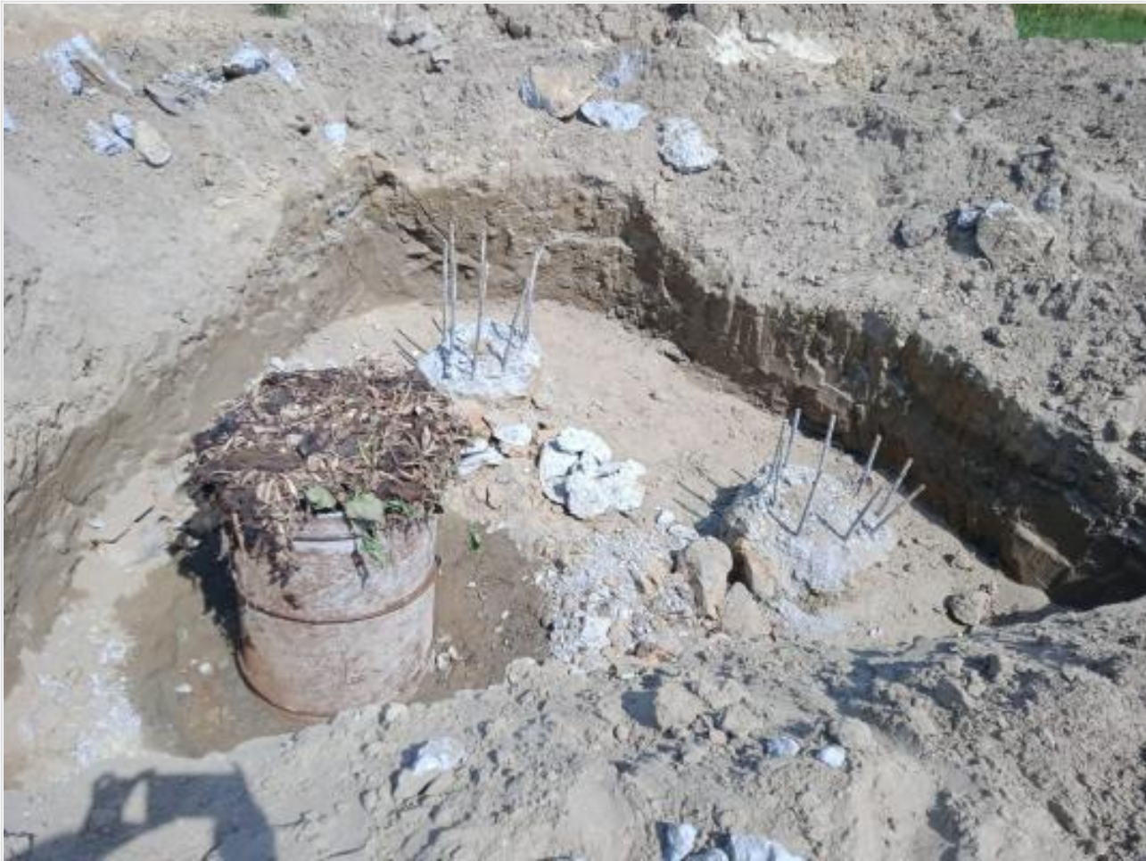
Pile head breaking on 10-05-23
