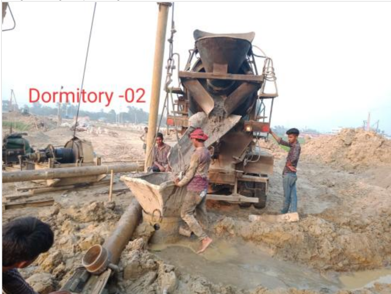
Ready mix concreting of pile on 25-03-23
