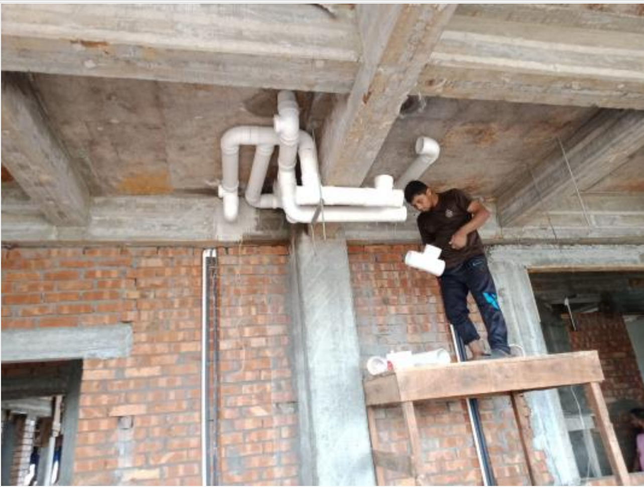
Comp. Bldg. Sanitary work on 29-08-23
