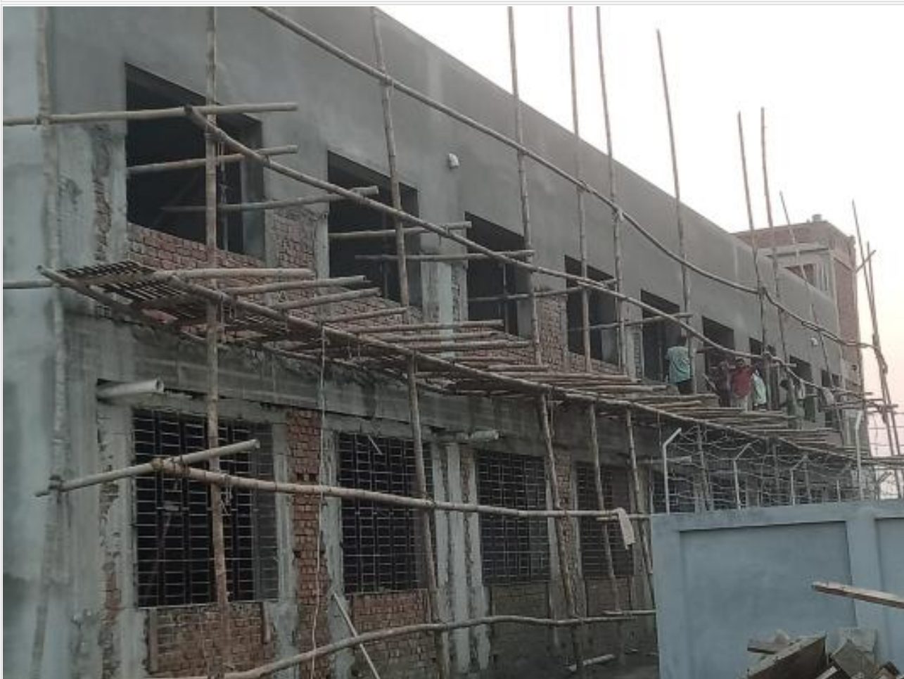
Comp. Bldg. Outside plaster work on 18-10-23
