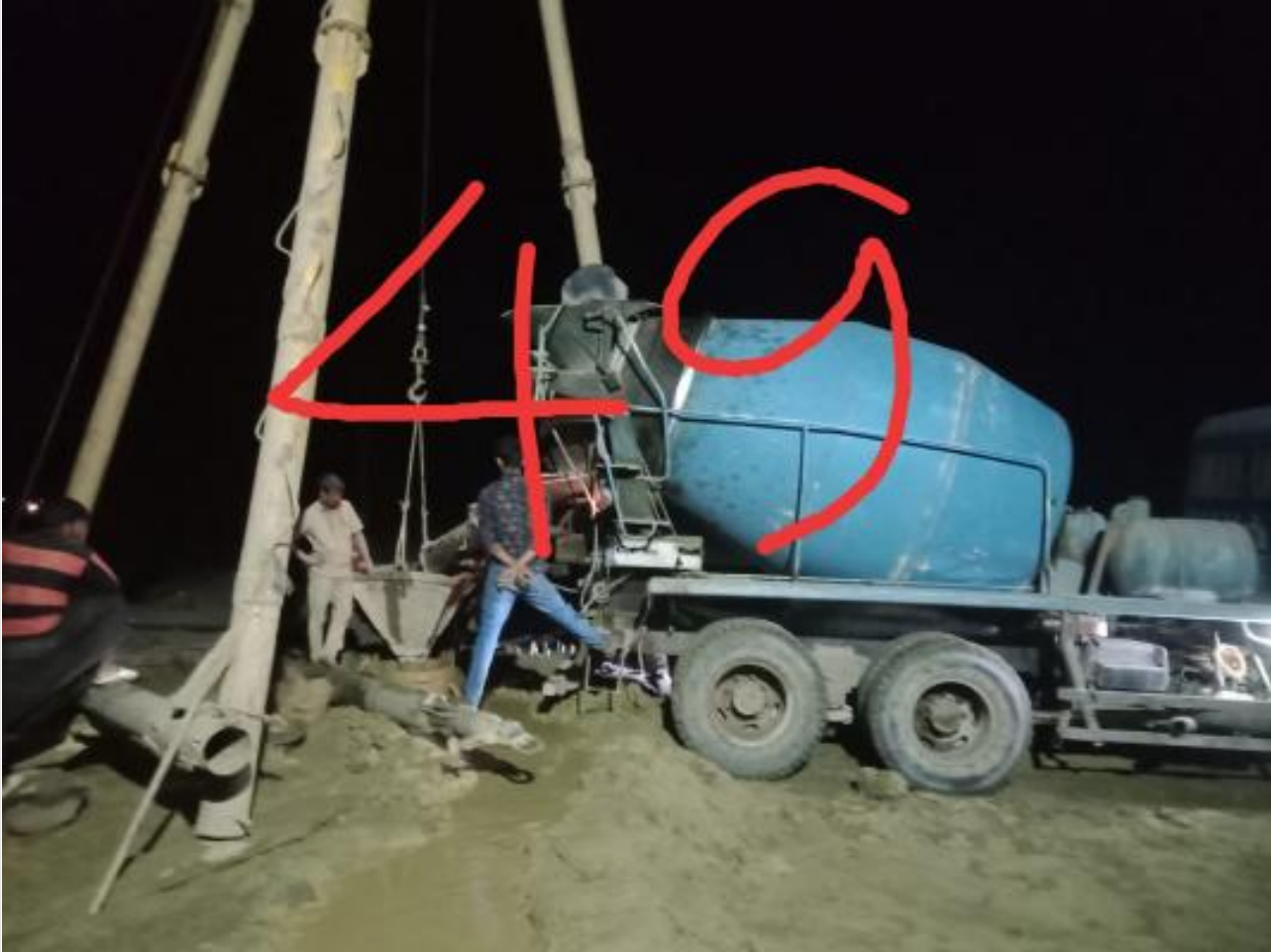
Ready mix concreting of pile on 08-03-23
