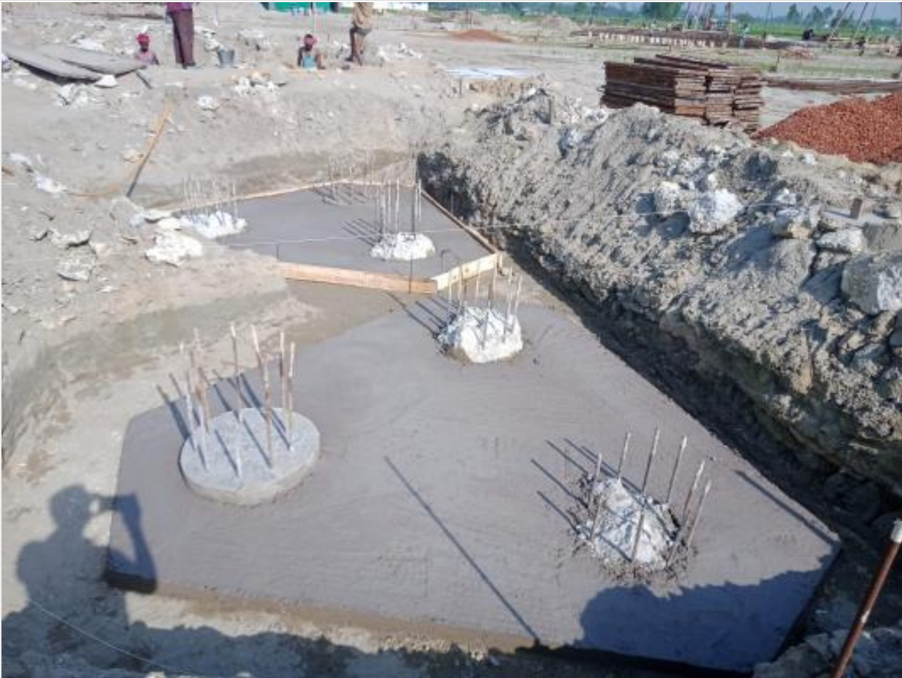
Pile cap CC work on 05-04-23
