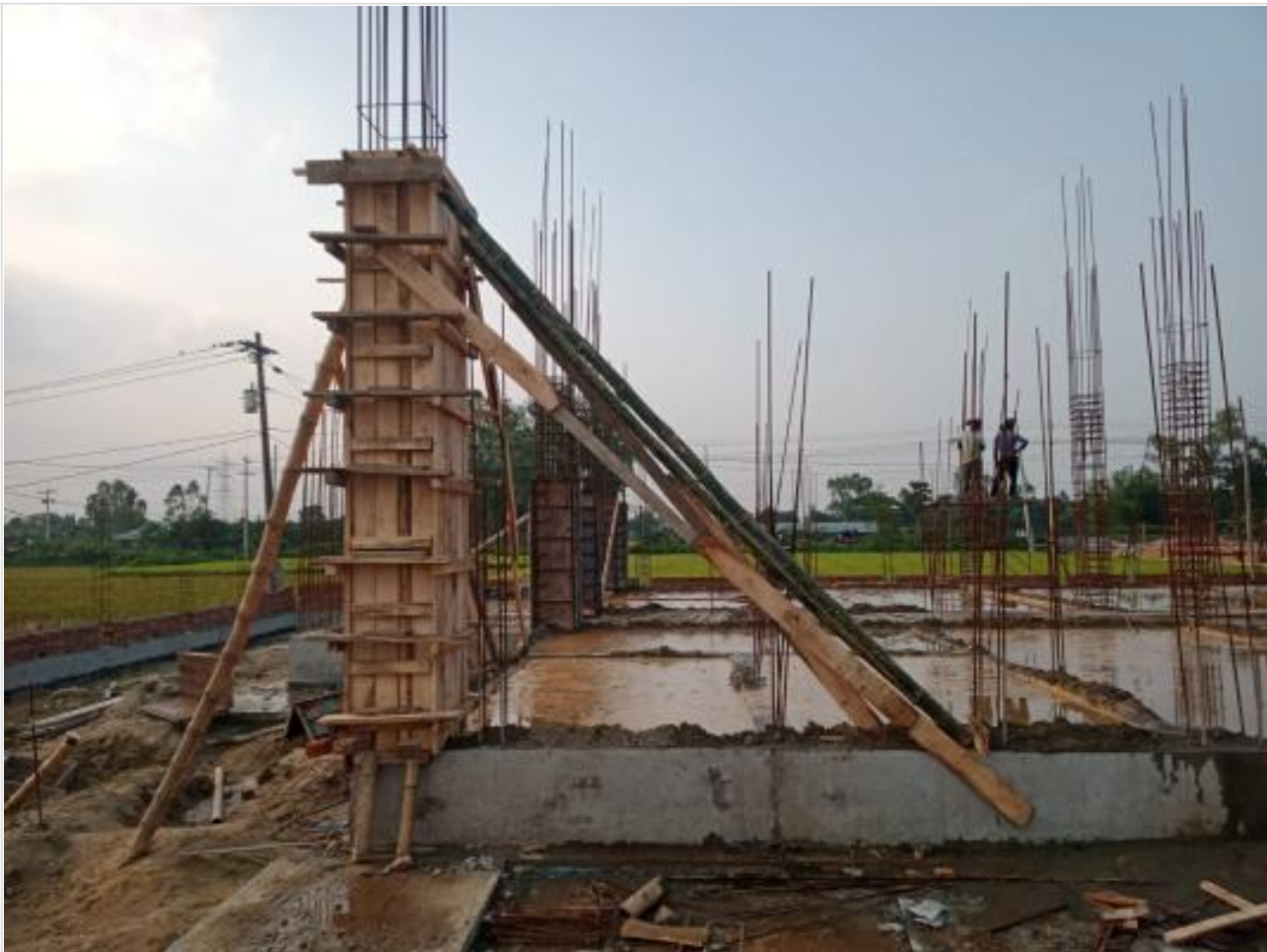
Comp. Bldg column shuttering on 26-05-23
