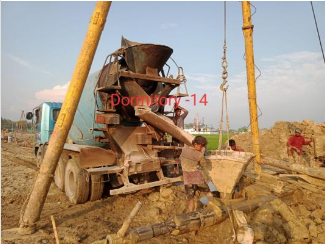
Ready mix concreting of pile on 01-04-23
