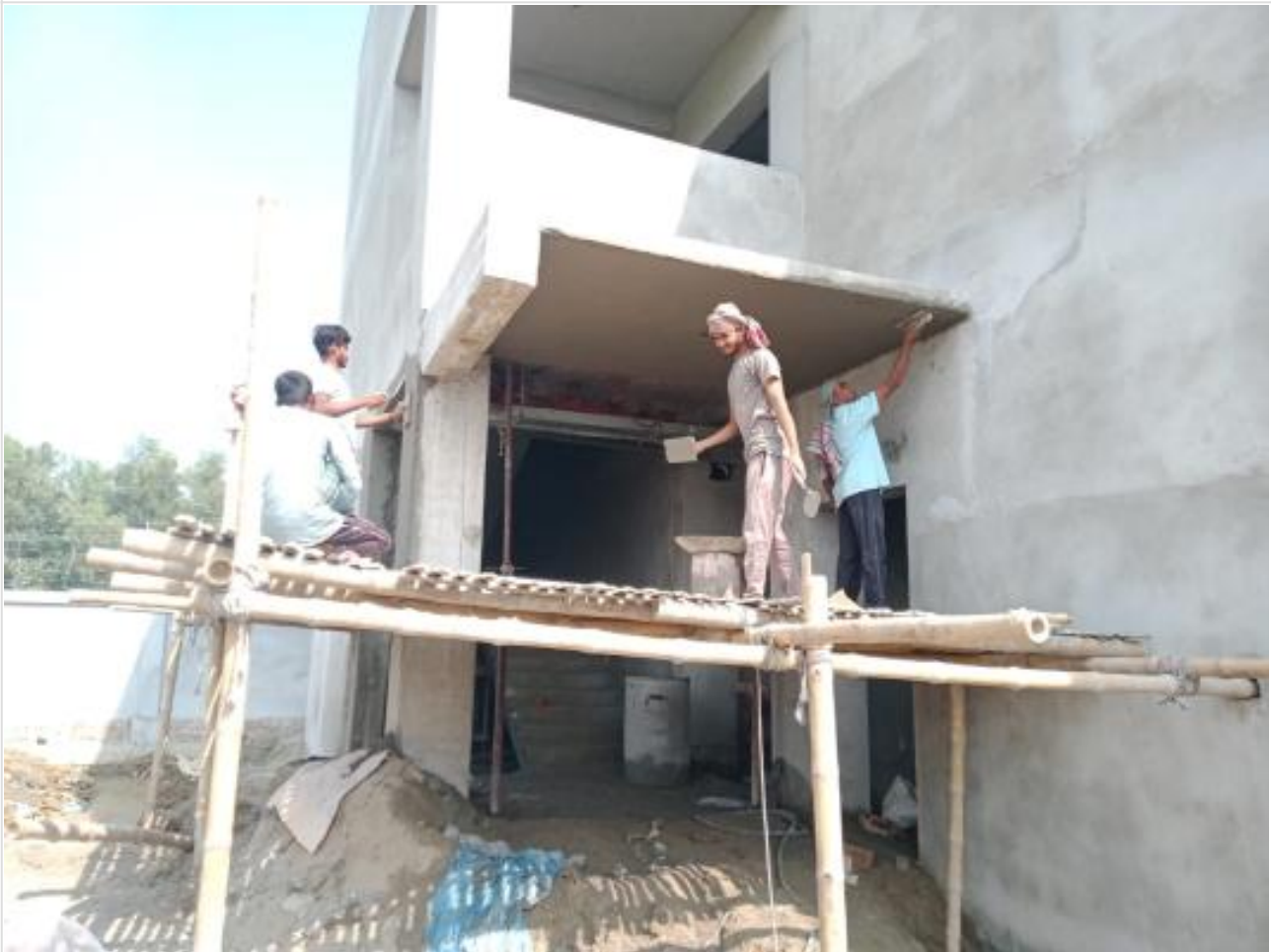
Dormitory canopy on 07-11-23
