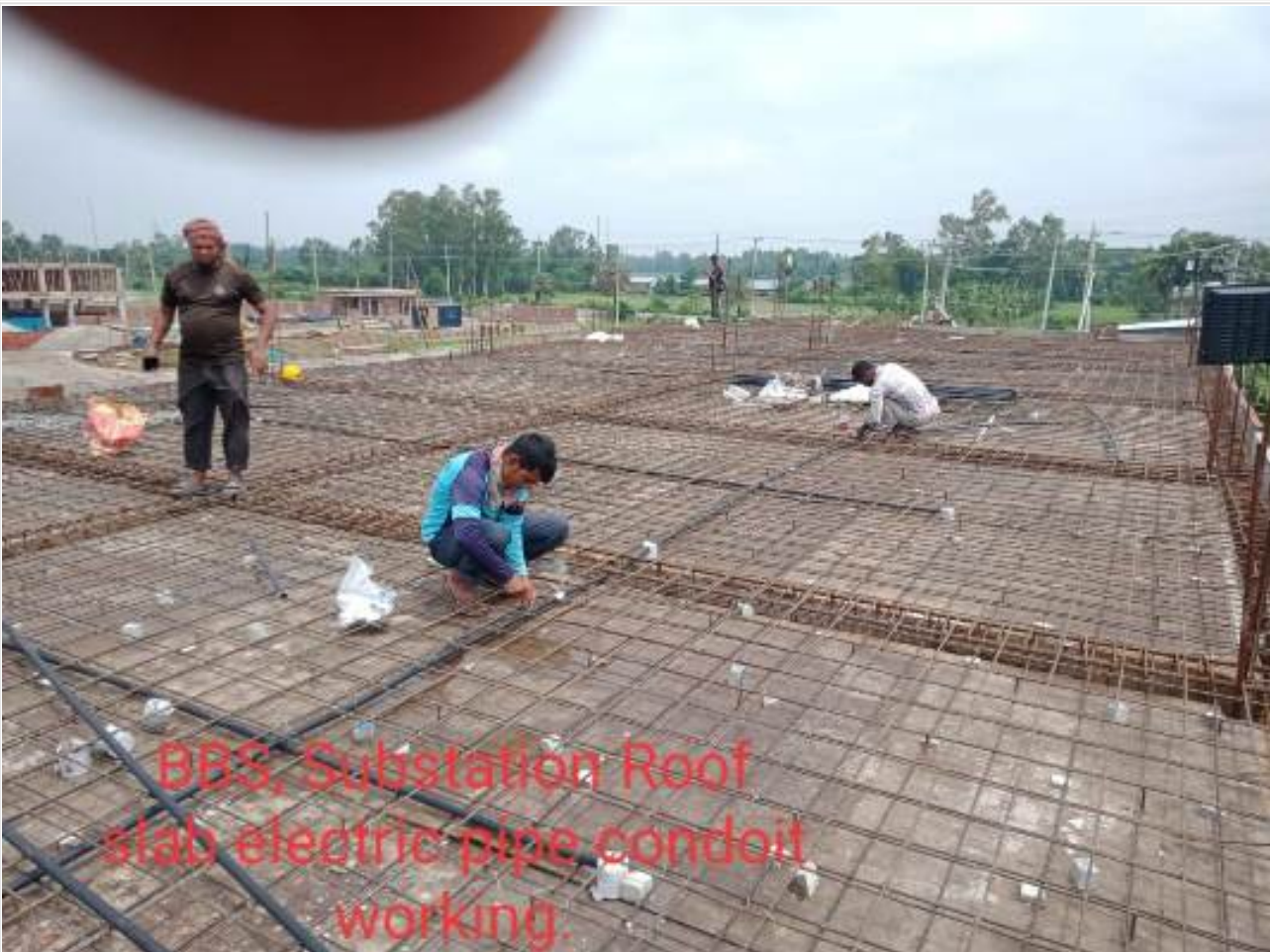
Sub-station-Electrical Pipe Work on 22-07-23
