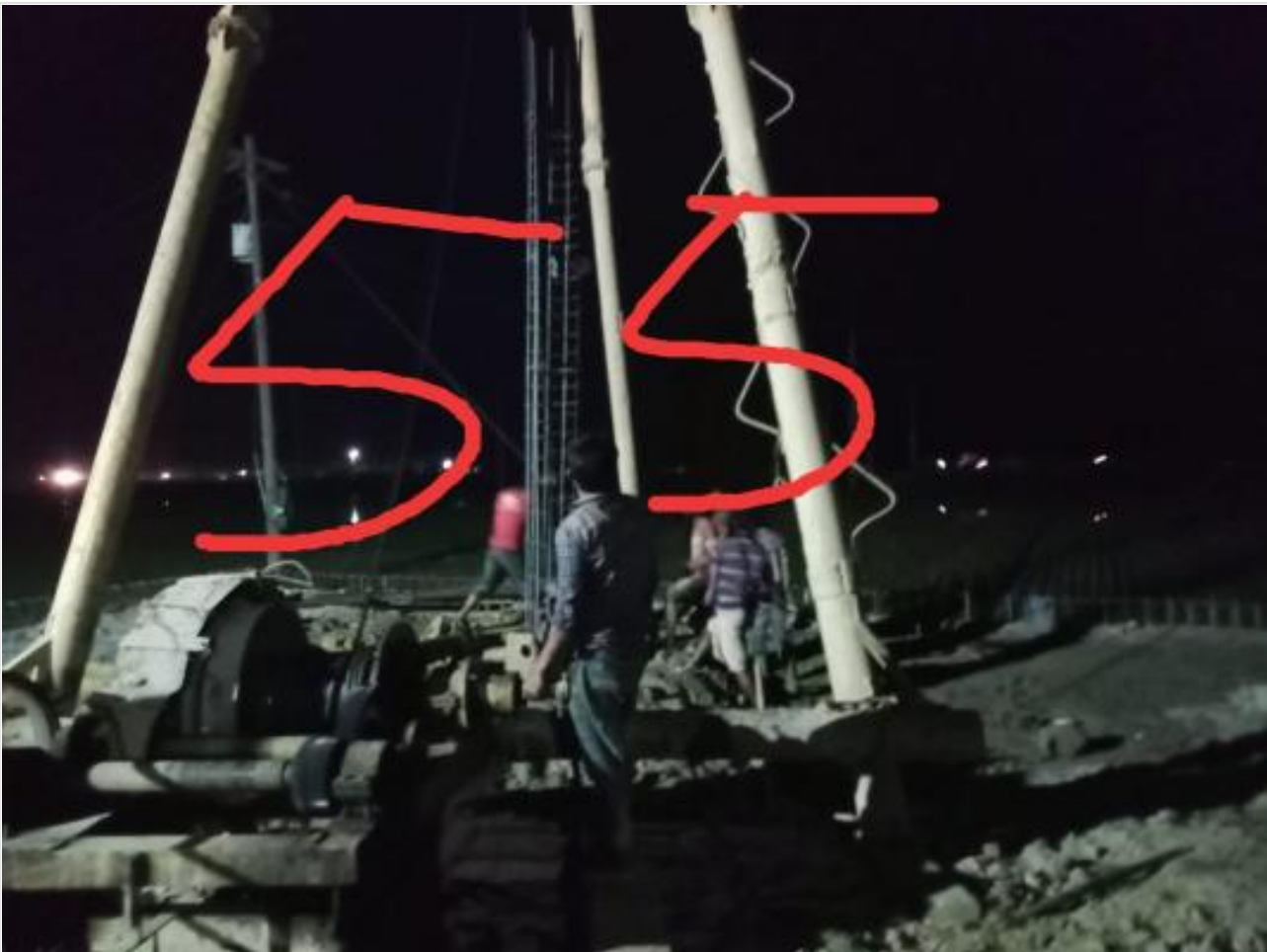
Ready mix concreting of pile on 10-03-23
