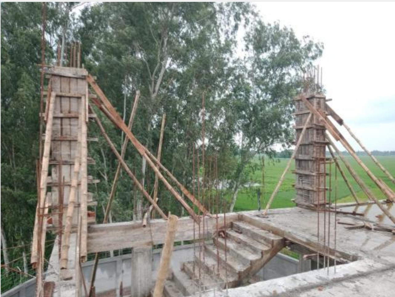
Dorm. Stair room column shuttering on 04-10-23
