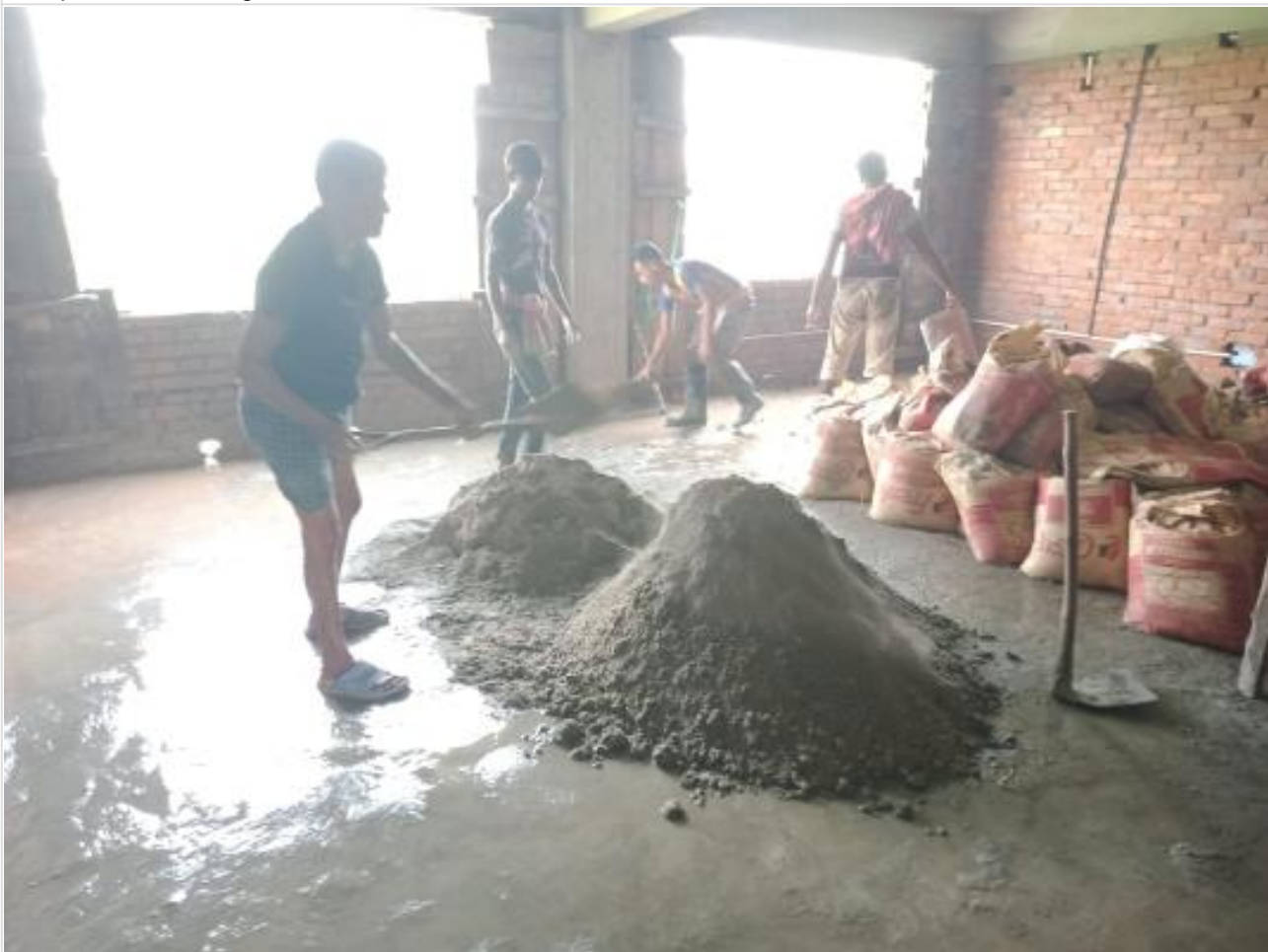
Comp. Bldg. GF casting on 29-09-23
