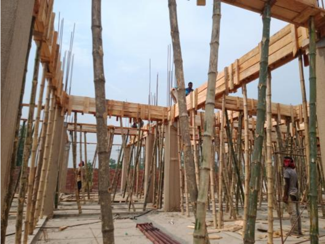
Comp. Bldg. Slab beam shuttering on 07-06-23
