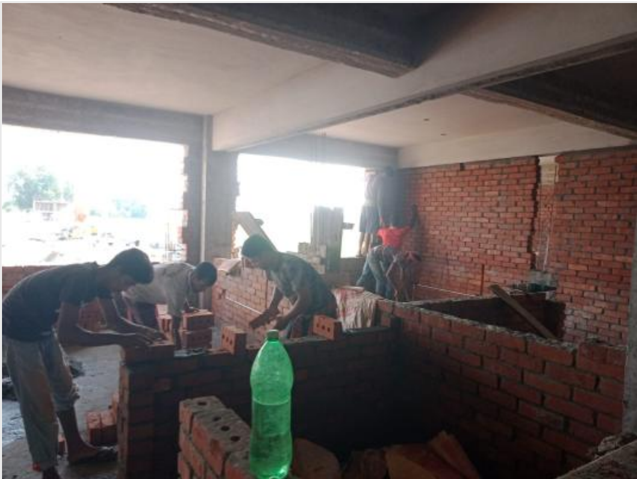
Comp. Bldg. FF Brick work on 09-09-23
