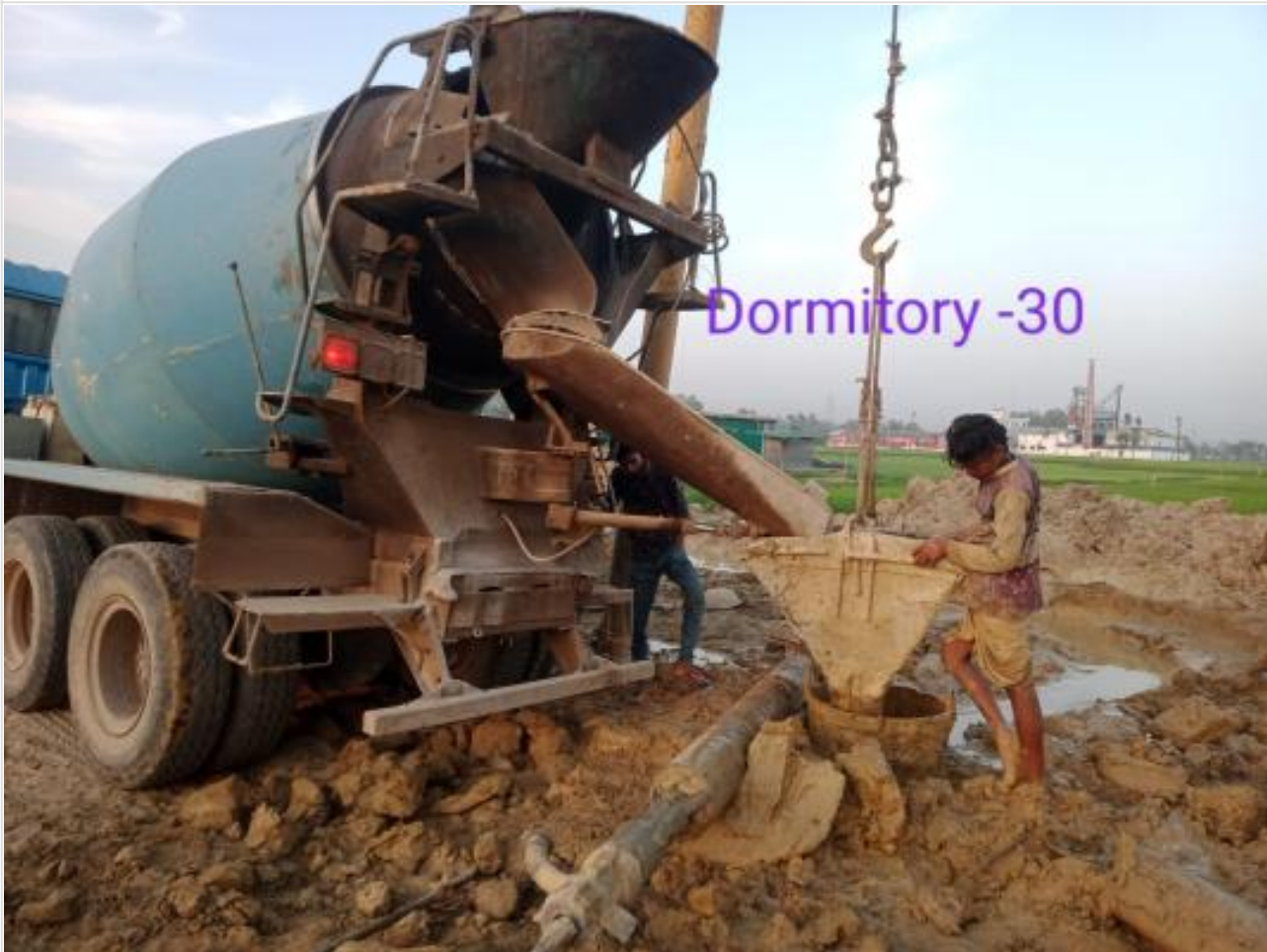
Ready mix concreting of pile on 08-04-23
