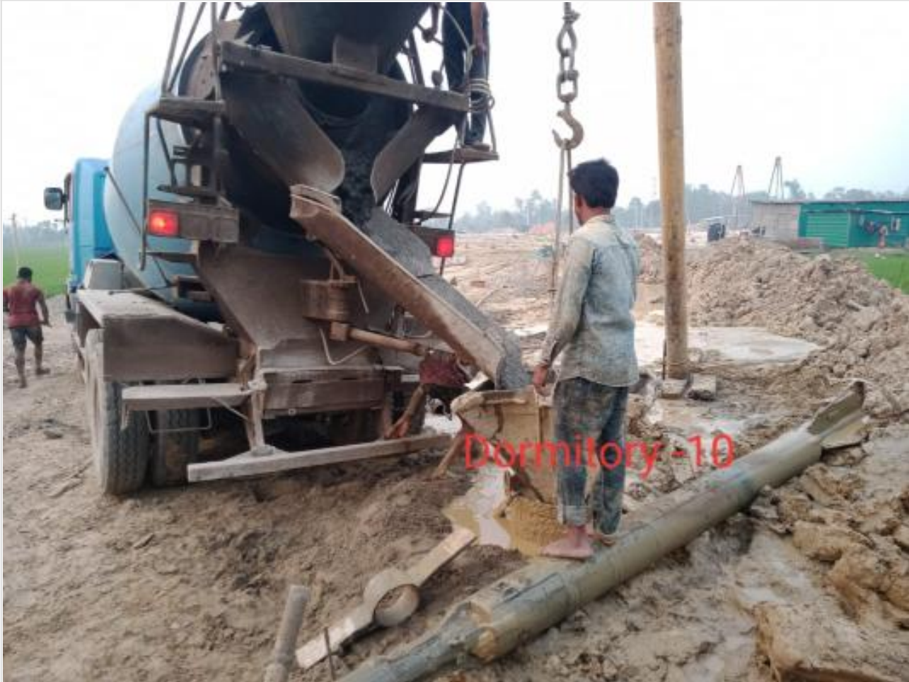
Dorm. Bldg. 10th pile concreting on 30-03-23
