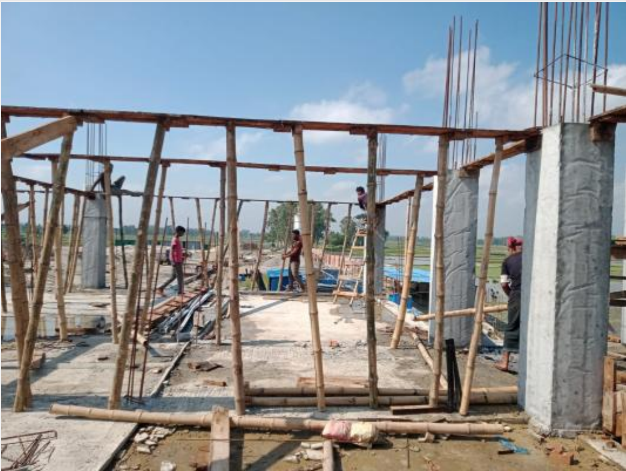
Comp. Bldg. 2nd Slab beam shuttering on 20-07-23
