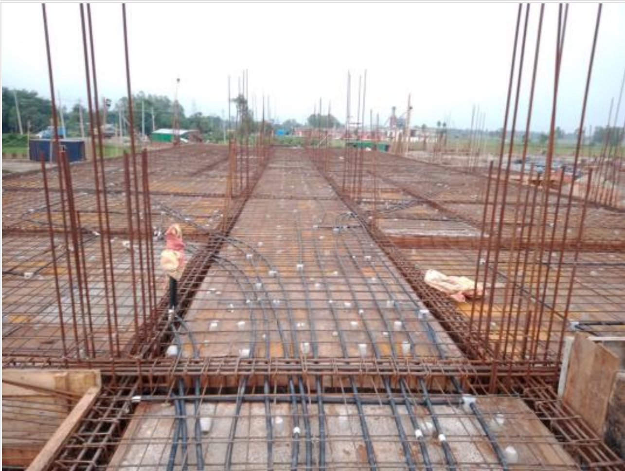
Comp. Bldg. Slab Ready for Concrete on 22-06-23
