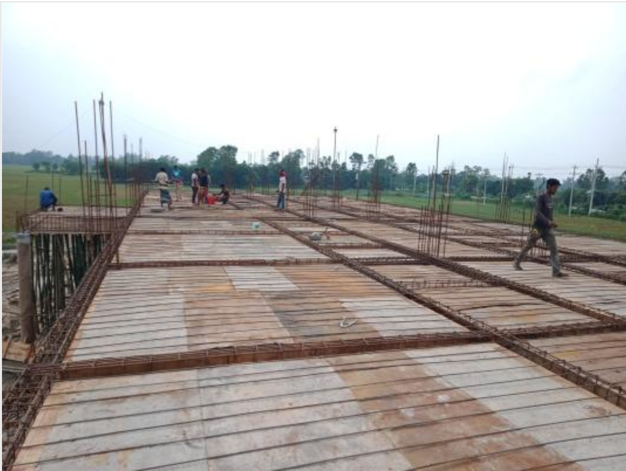
Comp. Bldg. Slab beam shuttering on 15-06-23
