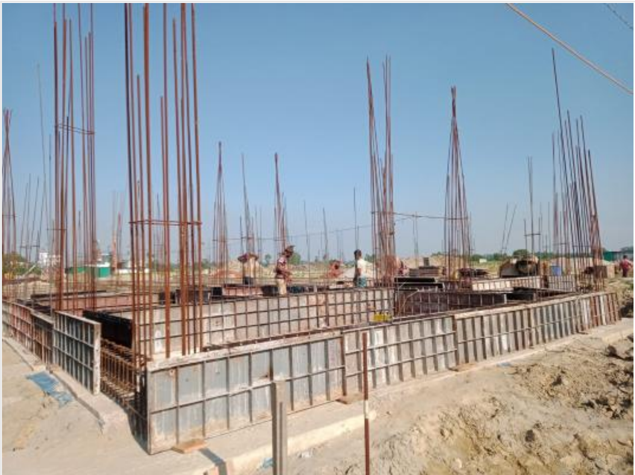
Comp. GB Shuttering on 06-05-23
