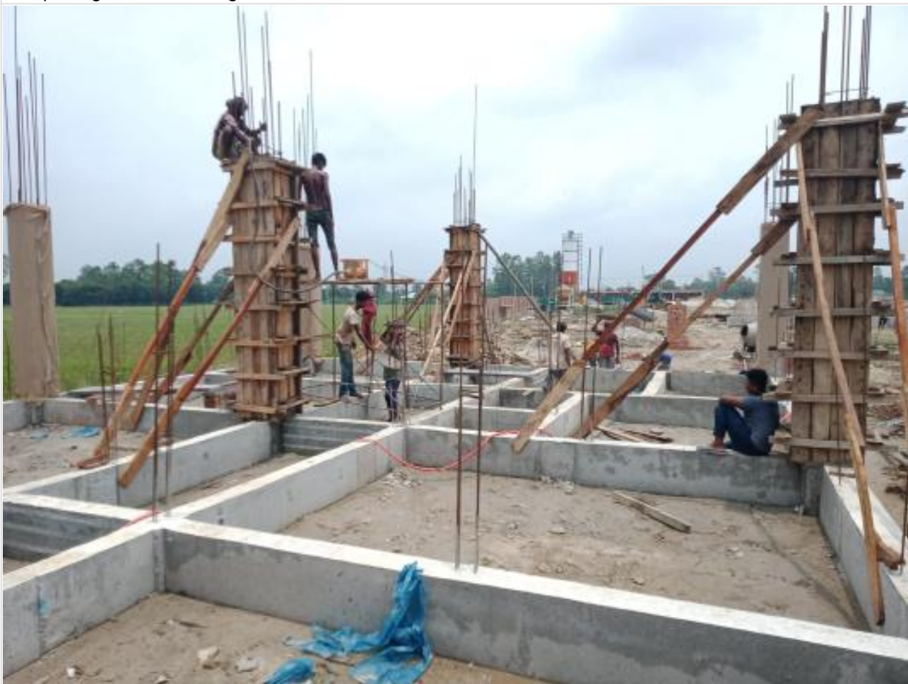
Dorm. Bldg. Column casting on 20-06-23
