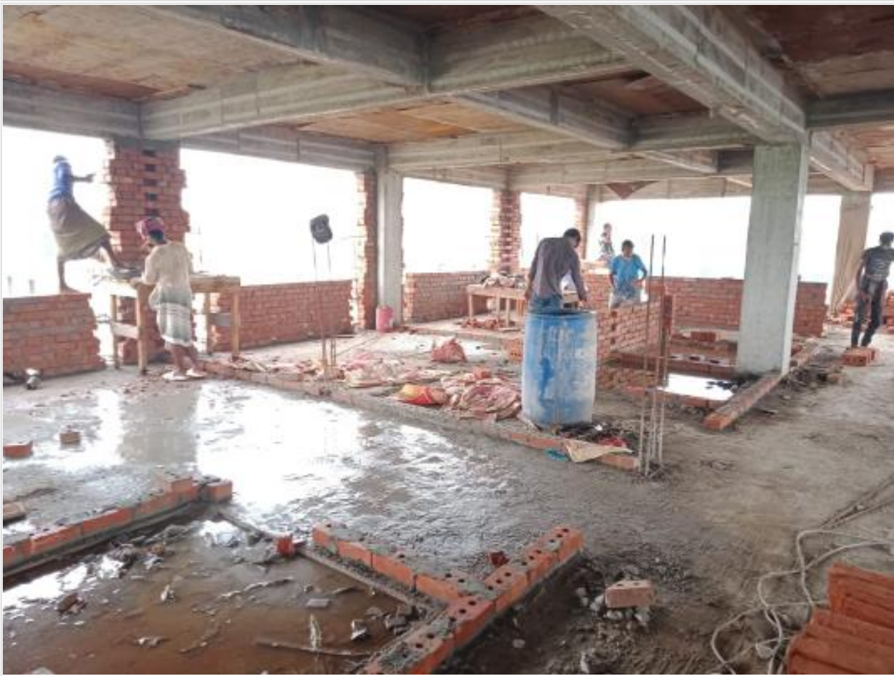
Comp. Bldg. 1st floor brick wall on 24-08-23
