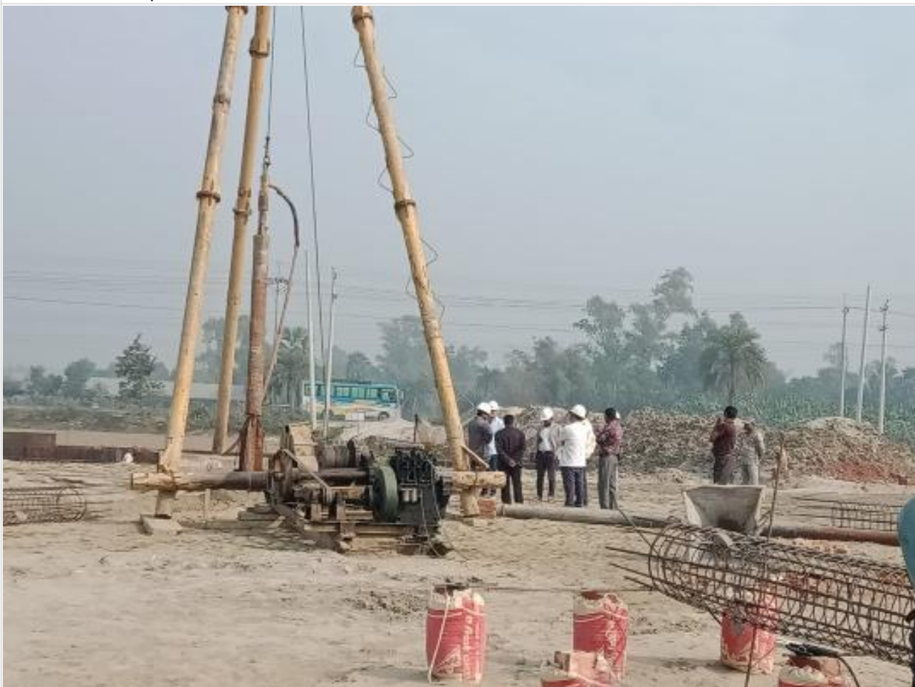
Inspection before Pile driving on 08-02-23
