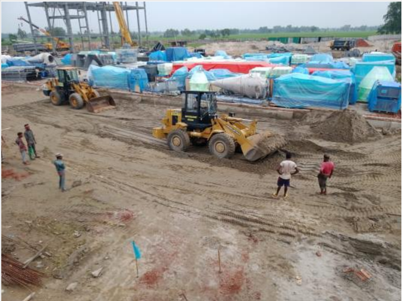
Road-Box cutting on 22-08-23
