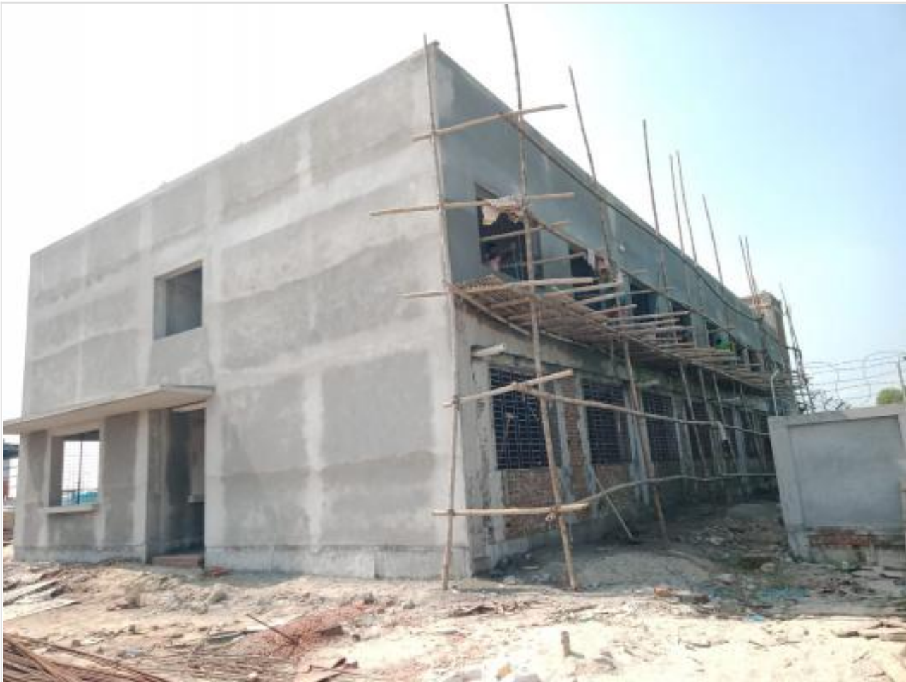
Comp. Building-Outside Plastering on 20-10-23
