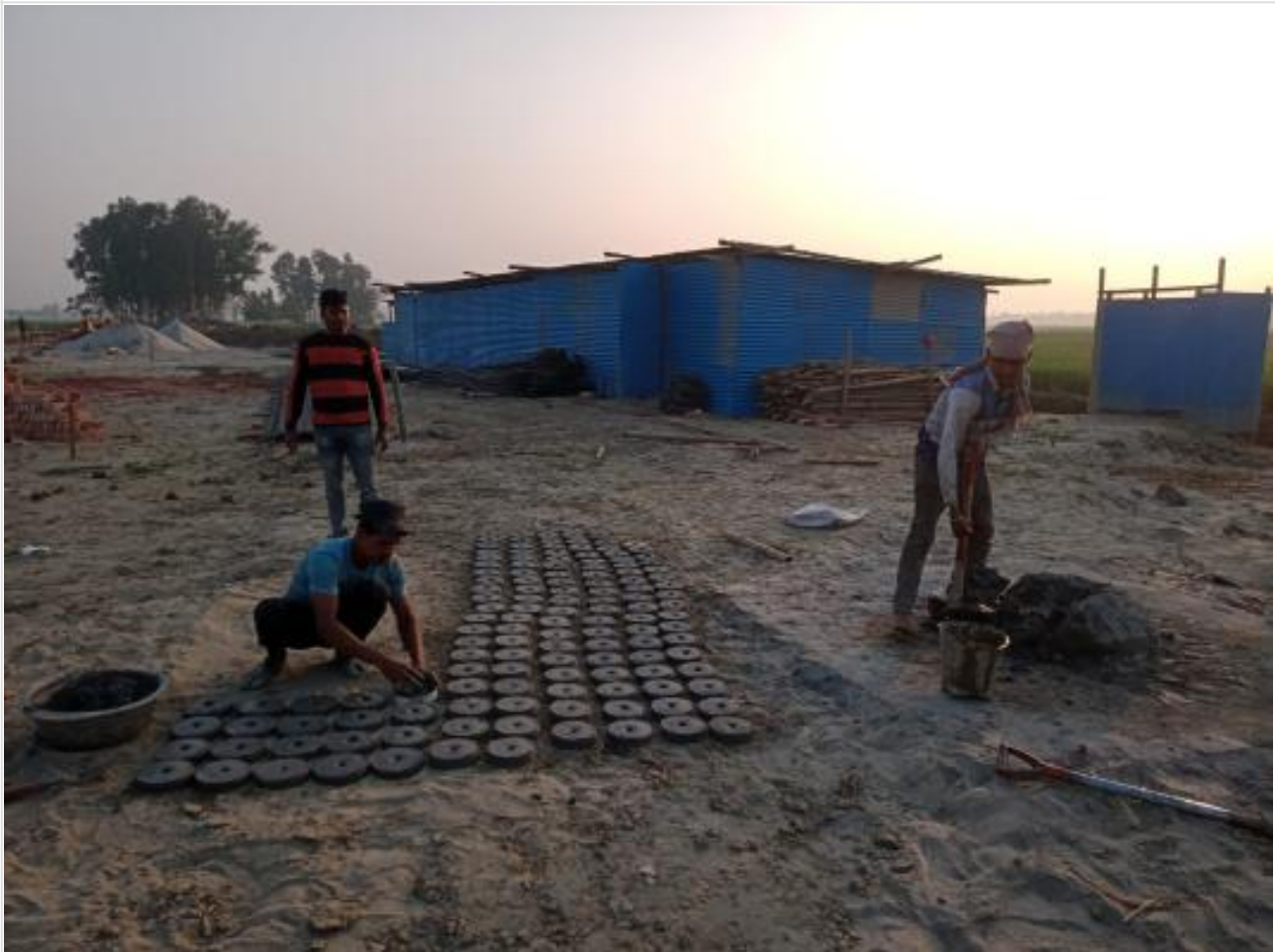
Pile re-bar spacer block making on 02-02-23
