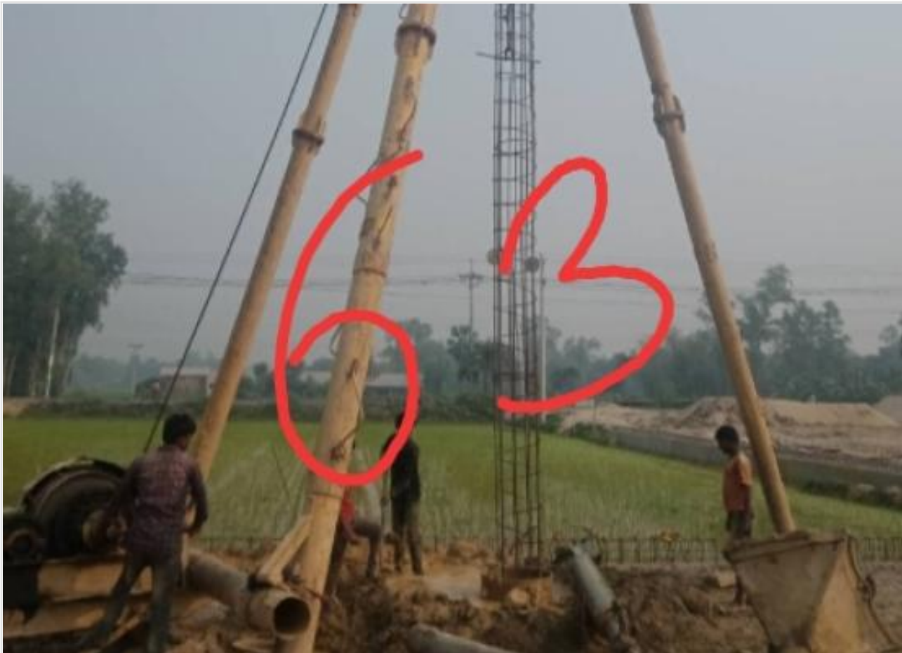
Com. Bldg. 63 Pile Boring on 14-03-23
