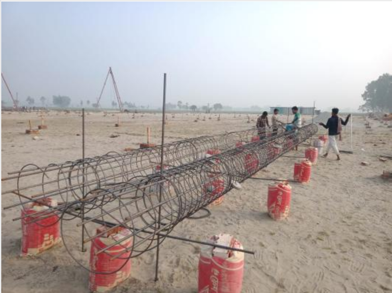
Pile Re-bar Work on 05-02-23
