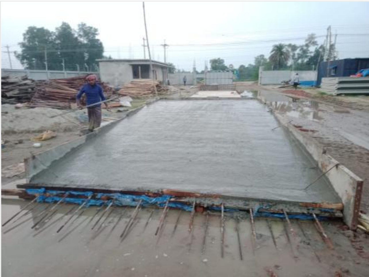
Weight scale concreting on 26-09-23
