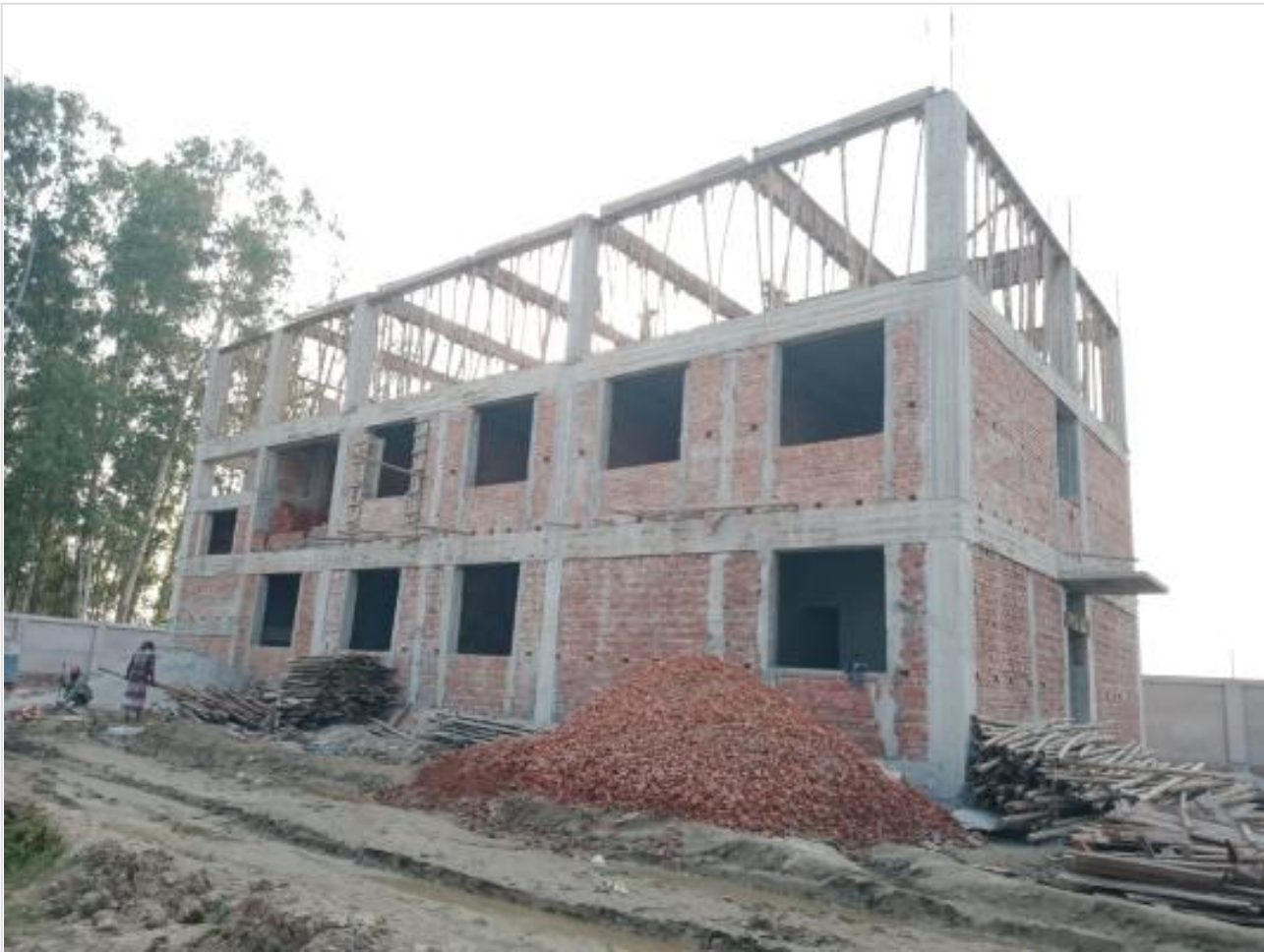
Dorm. Bldg. 2nd floor shuttering work on 06-11-23
