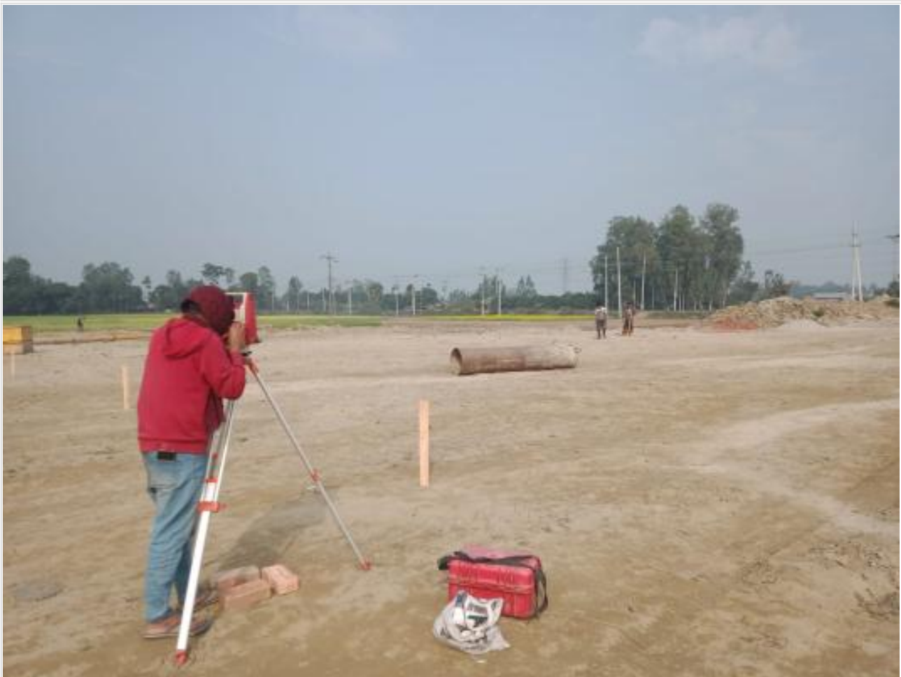
Pile Point Layout and Survey on 01-02-23
