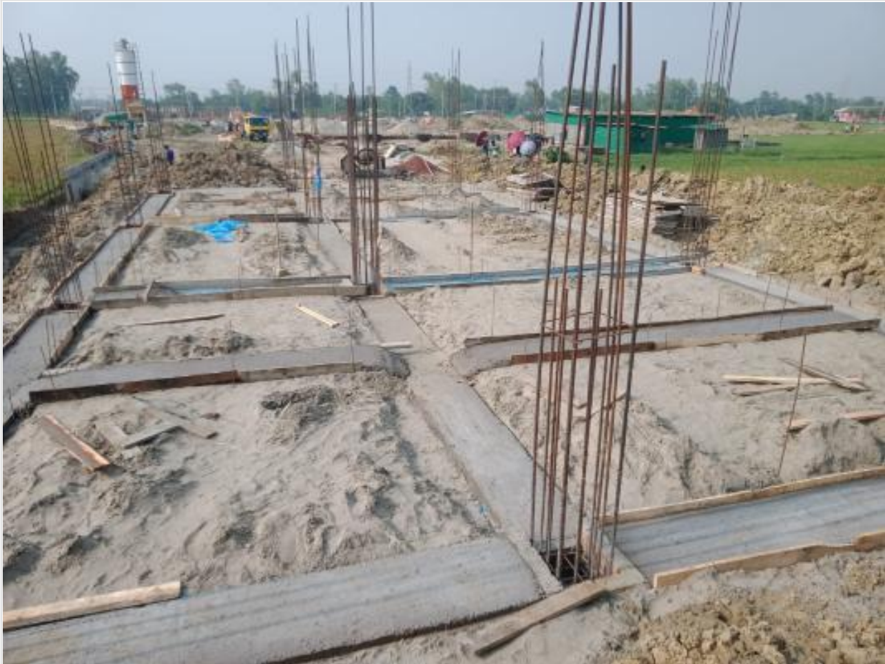
Dorm. Bldg. GB Bottom CC work on 03-06-23
