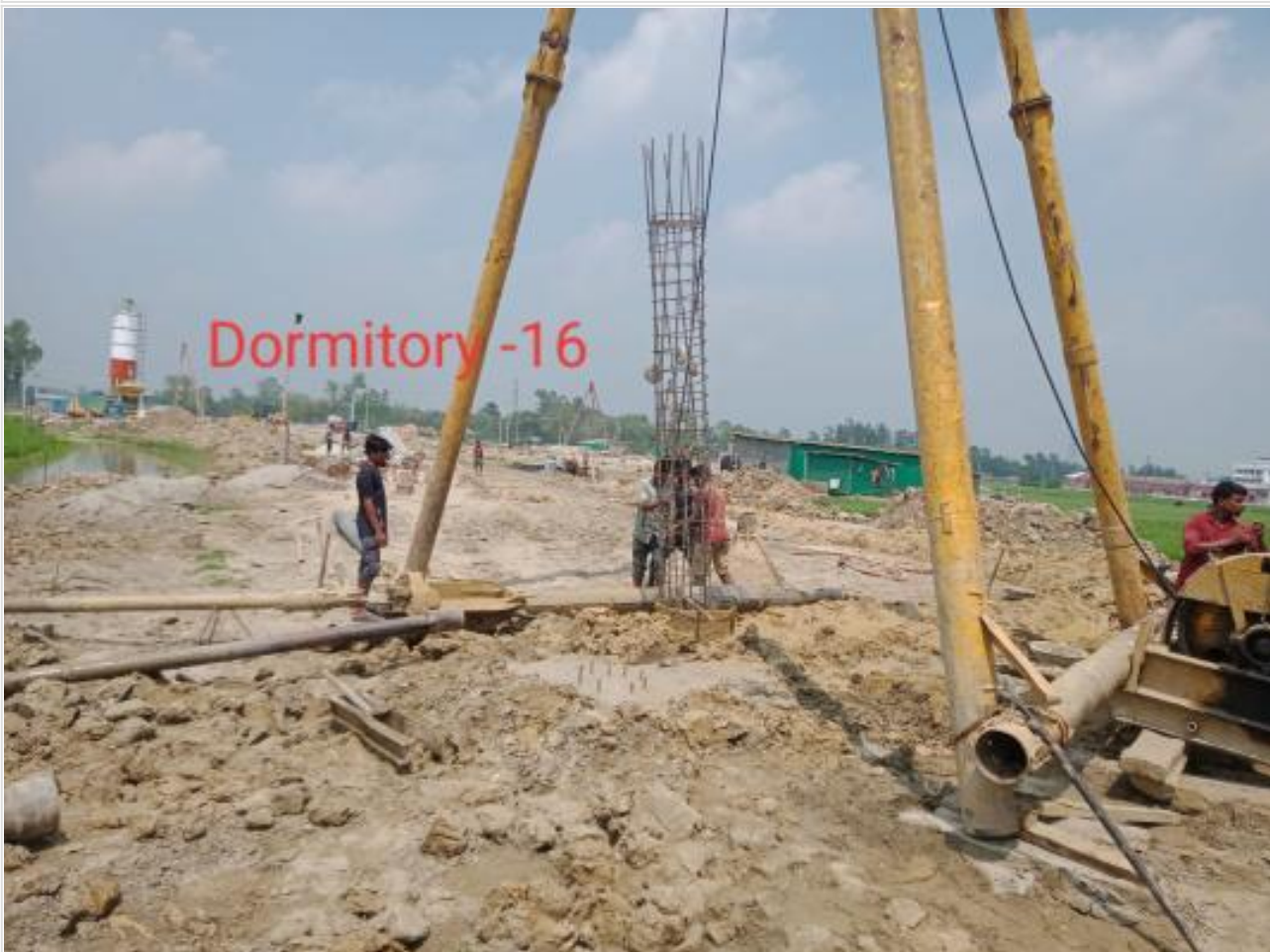
Ready mix concreting of pile on 01-04-23
