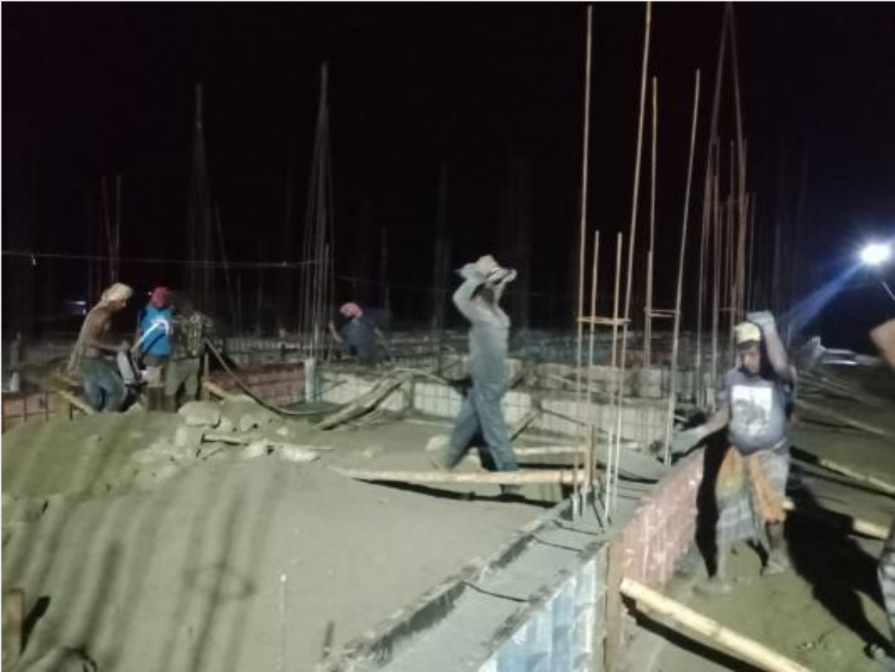
GB Concreting on 16-05-23
