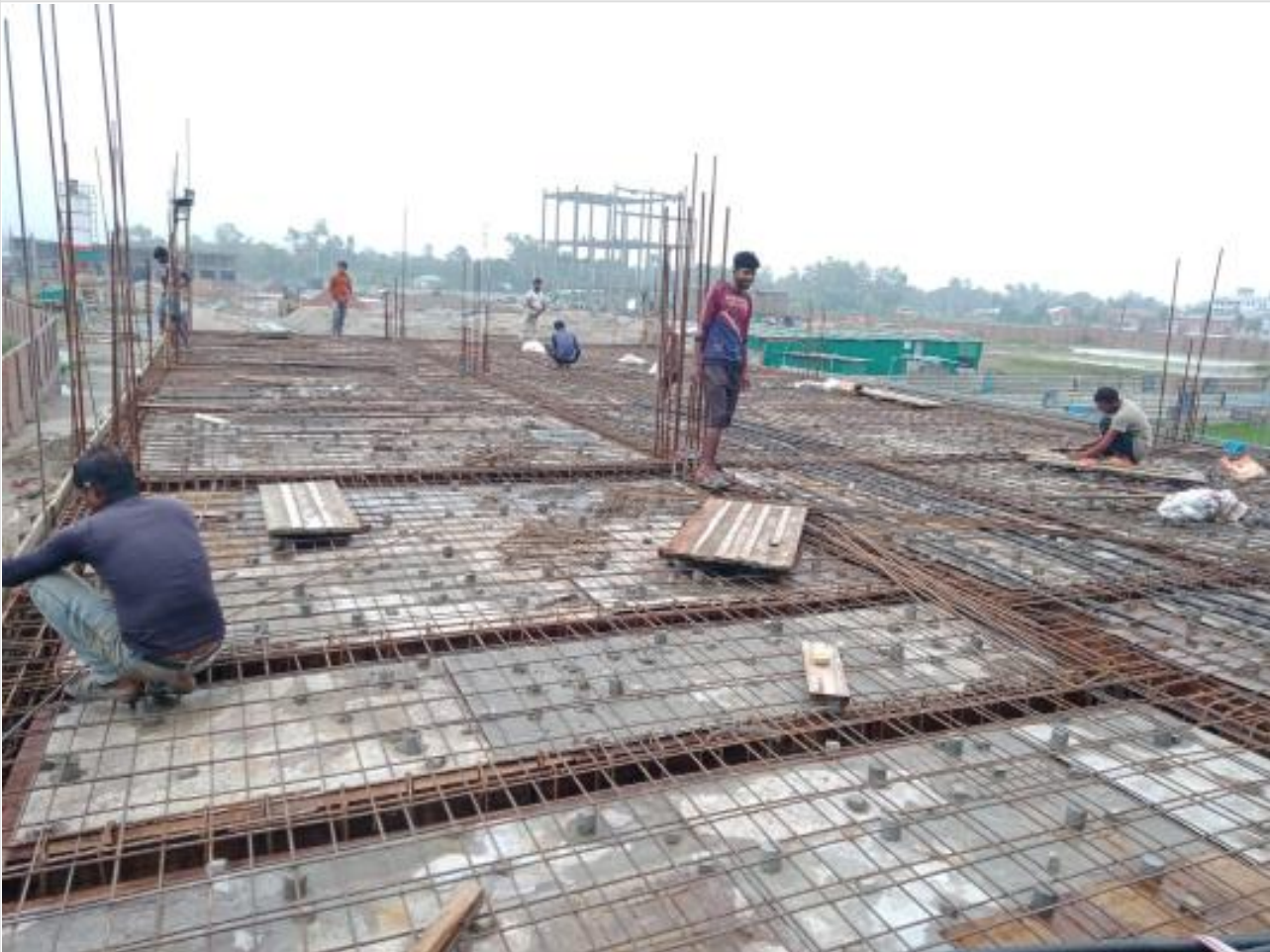
Dormitory Slab Electrical Pipe Laying on 08-08-23
