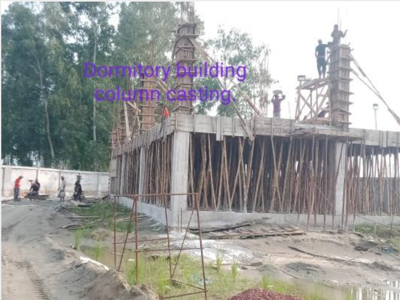
Dormitory Column Concreting on 23-08-23
