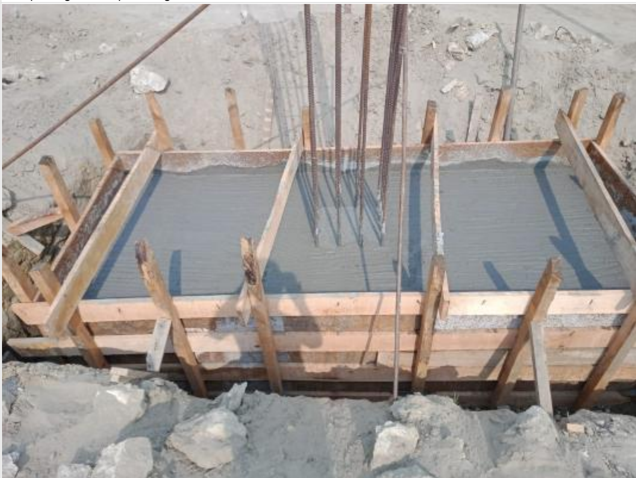
Pile Cap concreting. on 16-04-23
