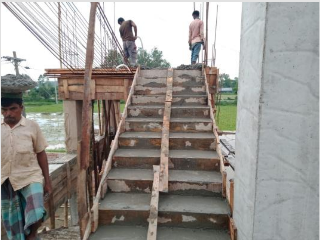
Comp. Bldg. 1st flight stair casting on 16-07-23
