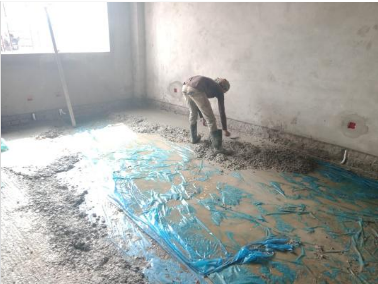
Comp. Bldg. GF casting on 09-10-23
