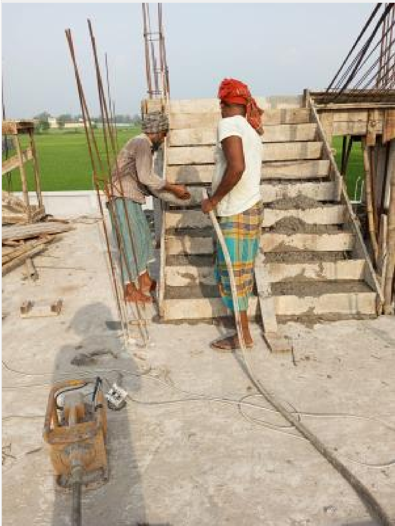
Dorm. Bldg. 1st flight stair casting on 30-08-23
