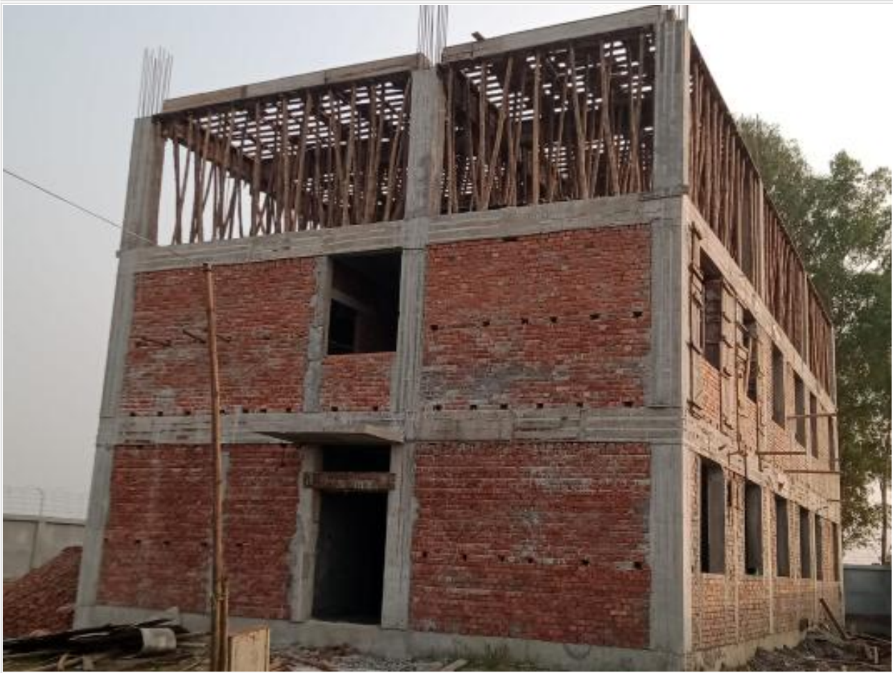
Dorm. Bldg. 3rd floor shuttering work on 09-11-23
