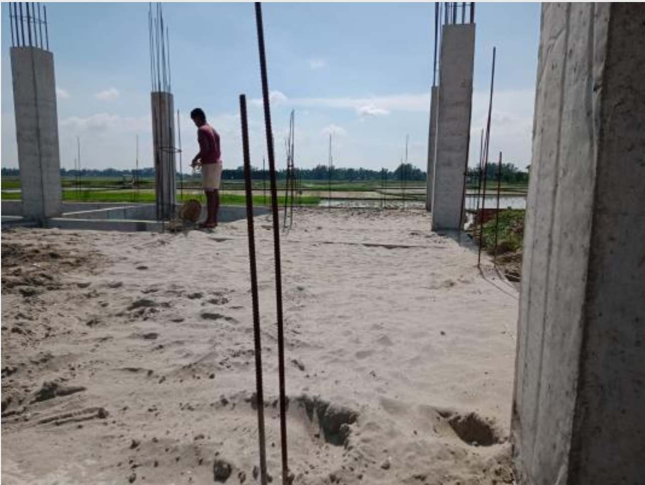
Dorm. Bldg. Sand filling on 18-07-23
