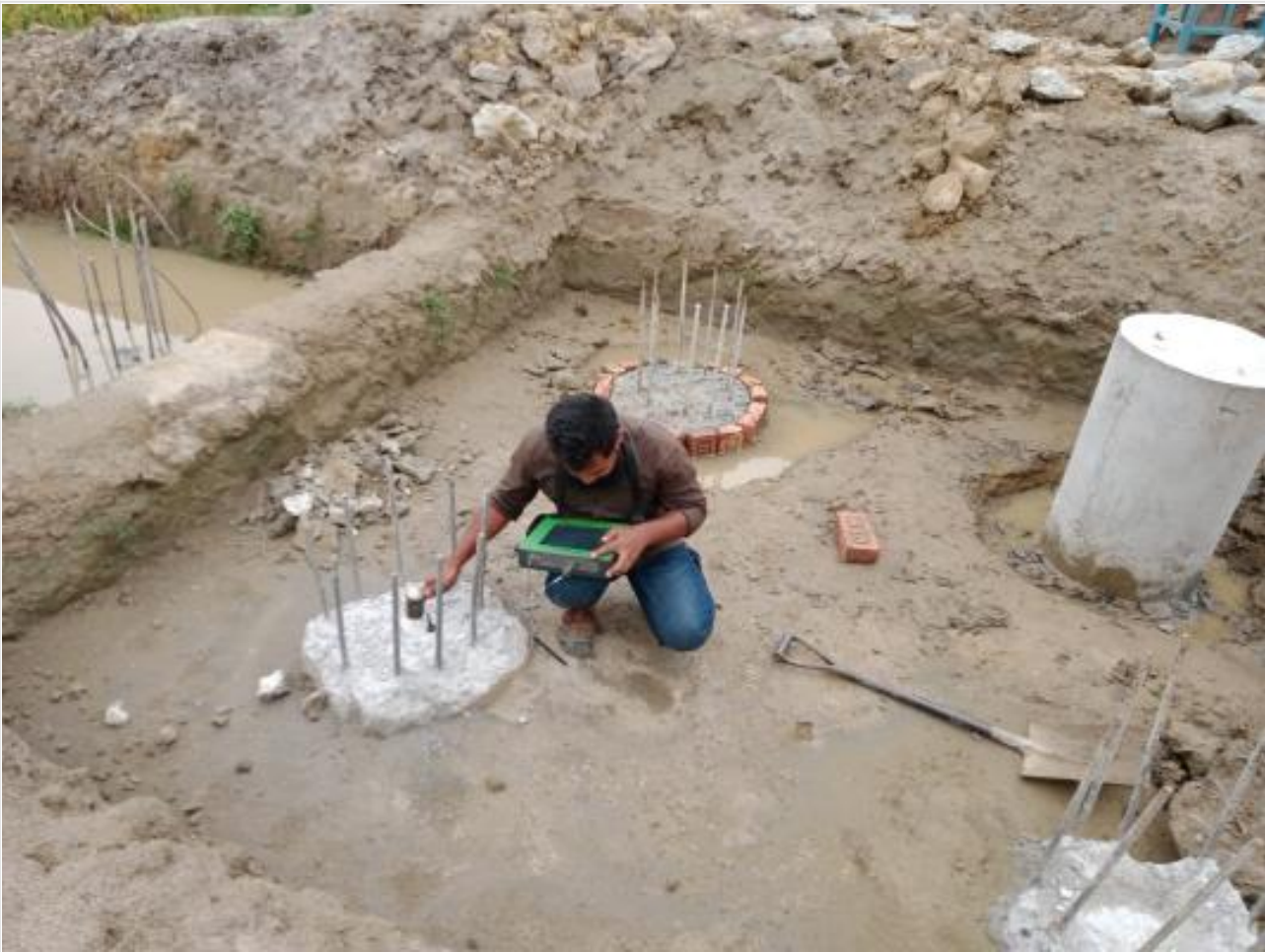
Pile integrity test on 19-05-23
