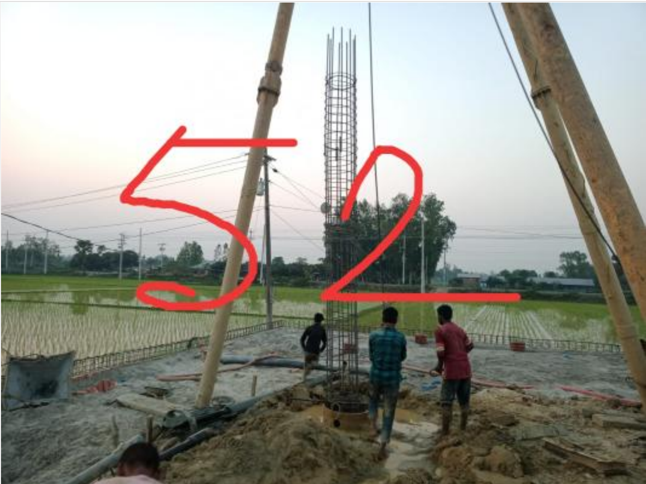
Ready mix concreting of pile on 09-03-23
