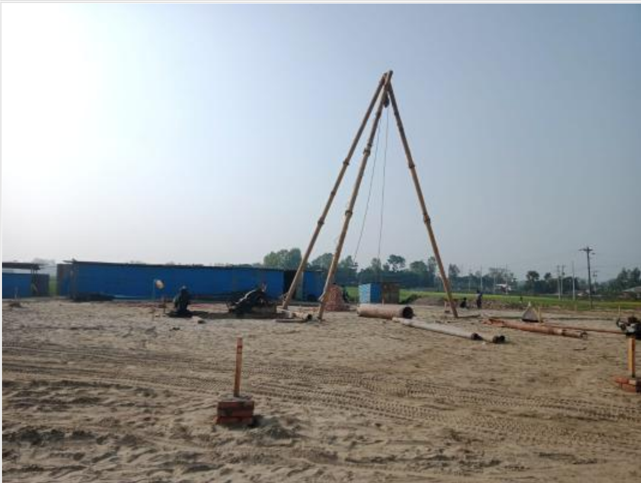
Pile Rig setting on 03-02-23
