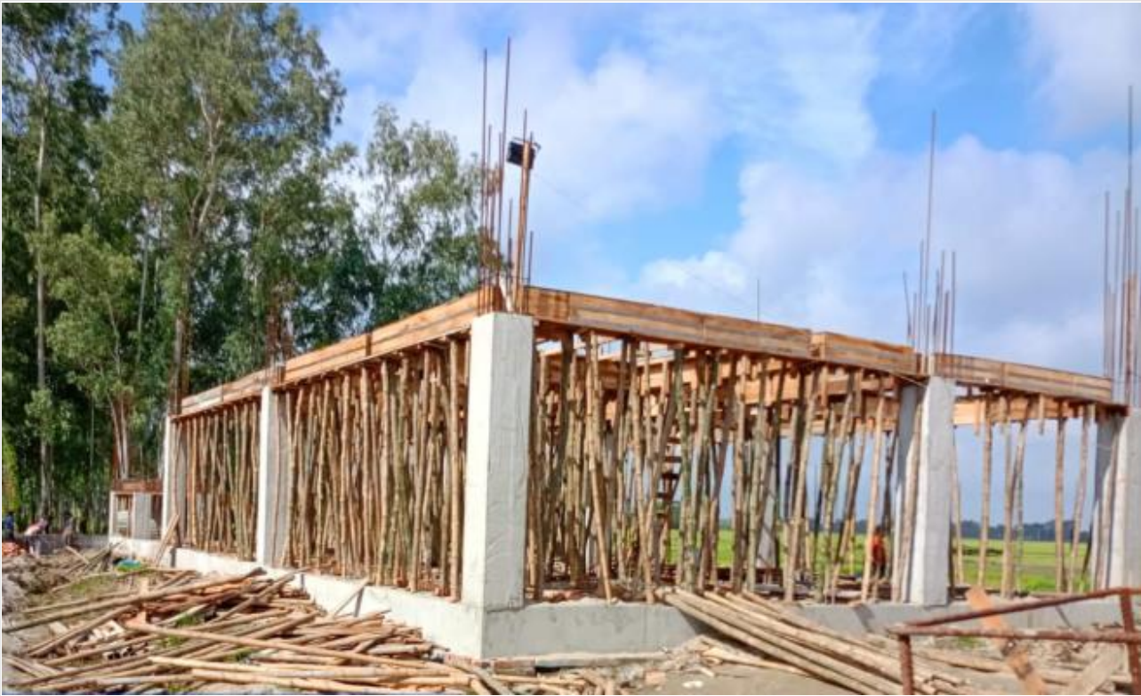
Dorm. Bldg shuttering work on 27-07-23
