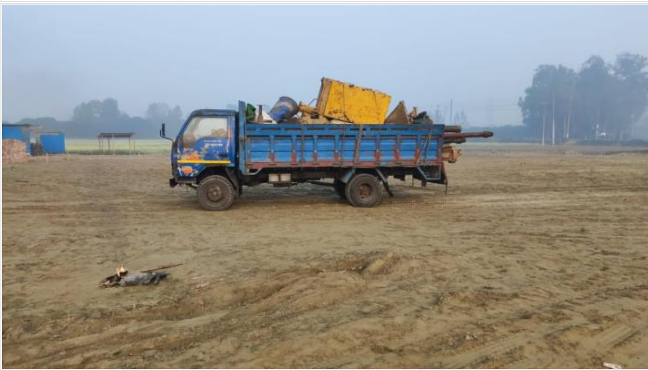
Piling Rig mobilized on 29-01-23
