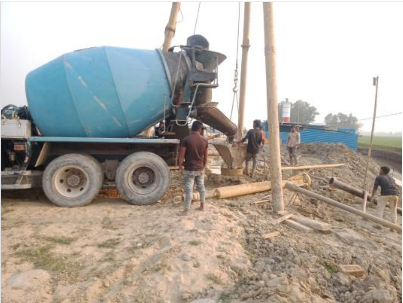
Ready mix concreting of pile on 16-02-23
