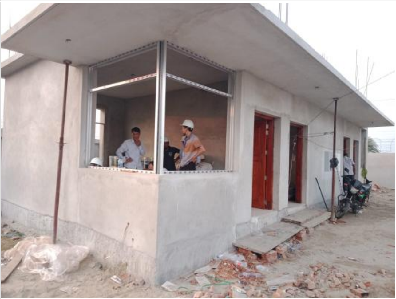
Gate House Thai work on 07-11-23
