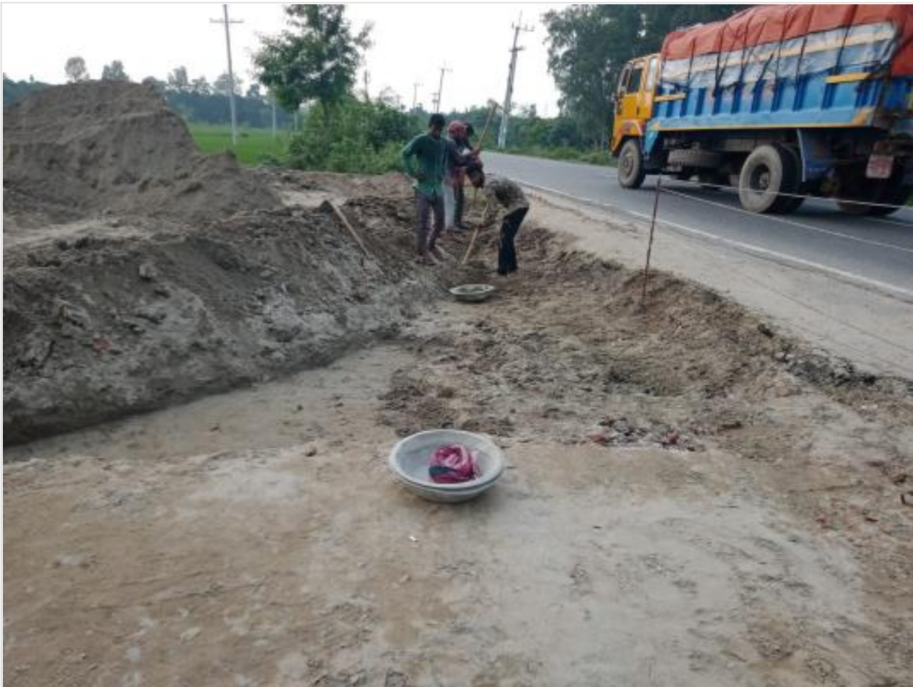
Road work on 11-10-23
