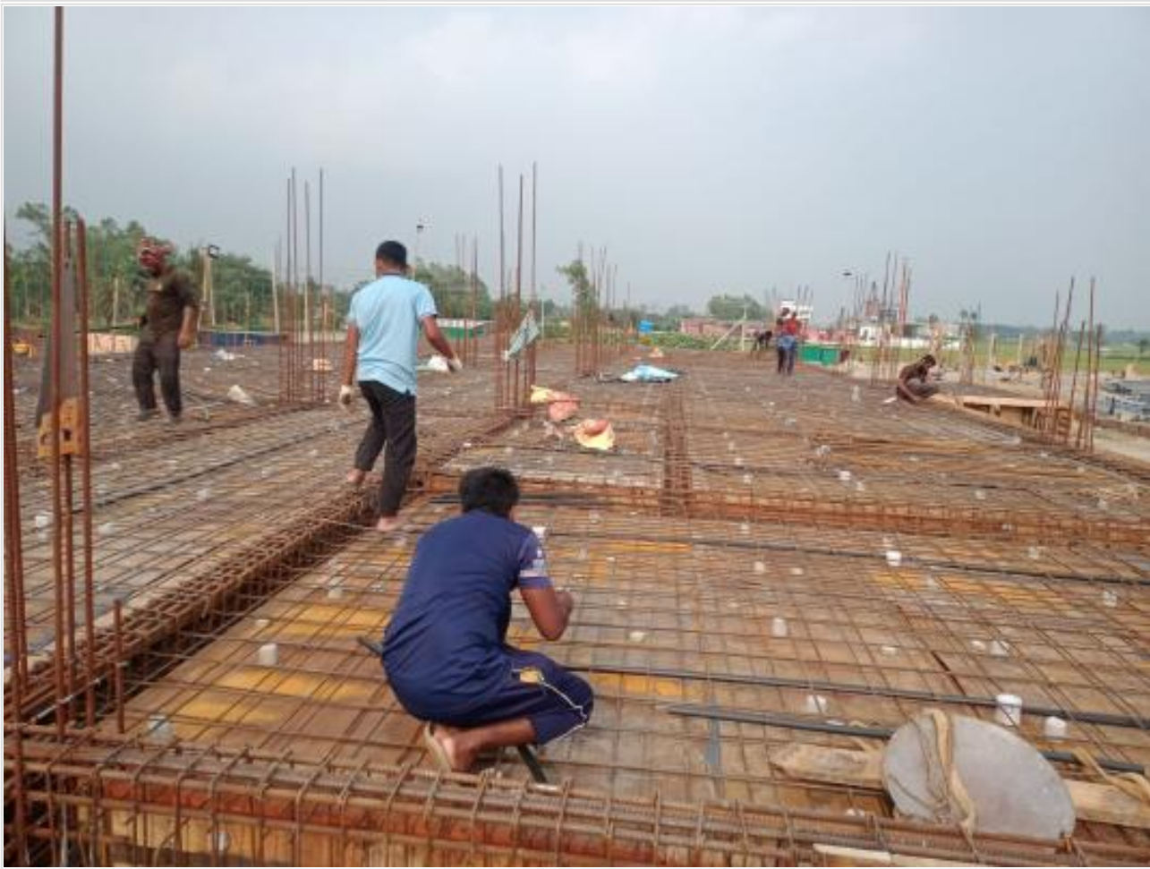
Comp. Bldg. Slab shuttering and Rod bind on 20-06-23
