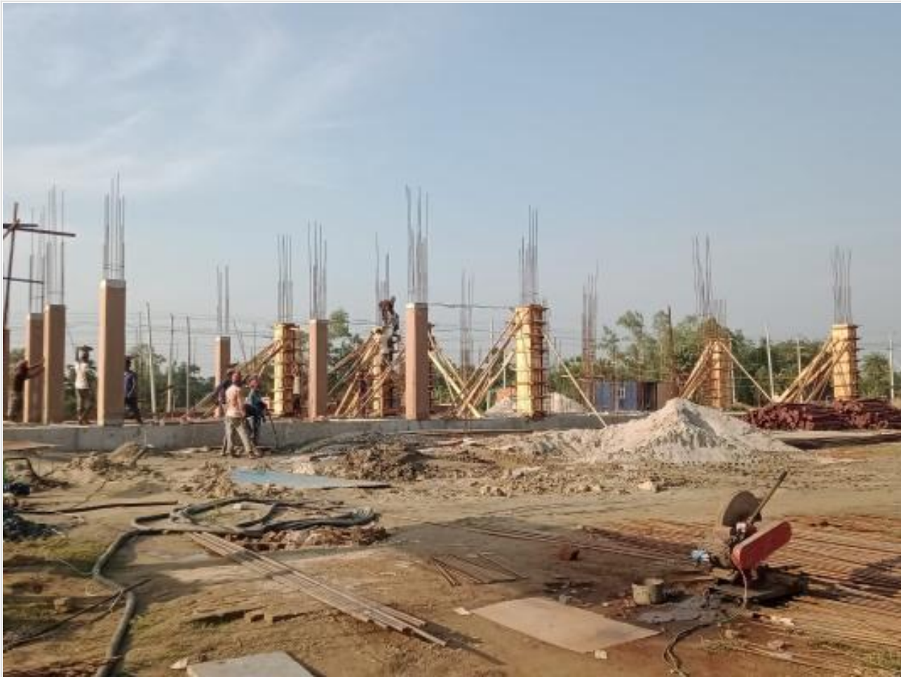
Comp. Bldg. Column shutter on 31-05-23
