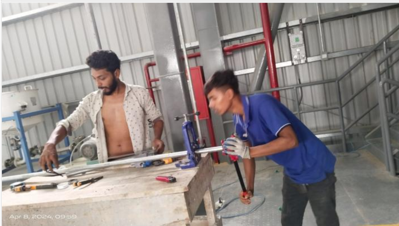
Electrical Work on 08-04-24
