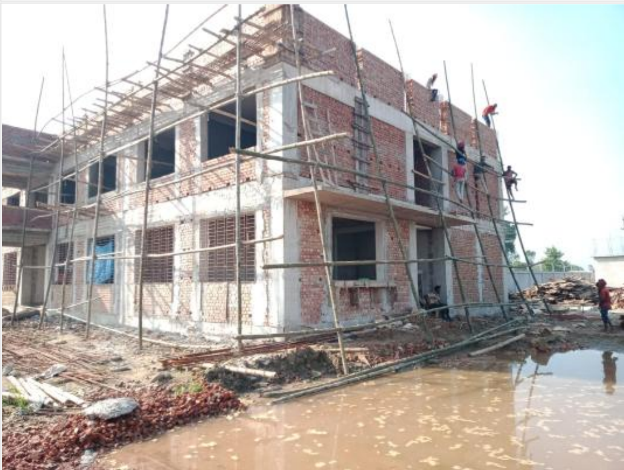
Comp. Bldg outside scaffolding on 28-09-23
