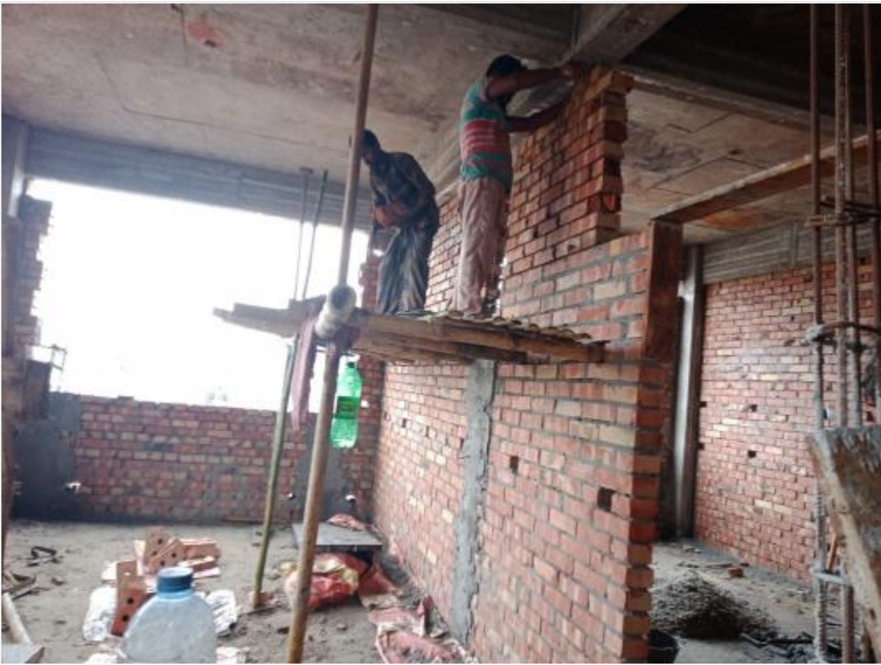
Comp-GF-Brick Work on 07-08-23
