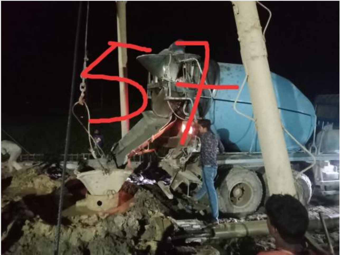
Ready mix concreting of pile on 12-03-23
