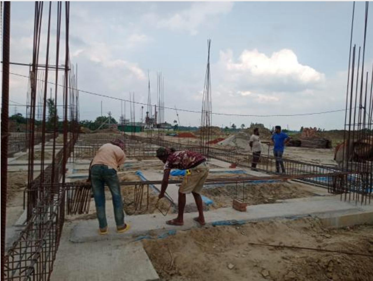
GB Re-bar work on 04-05-23
