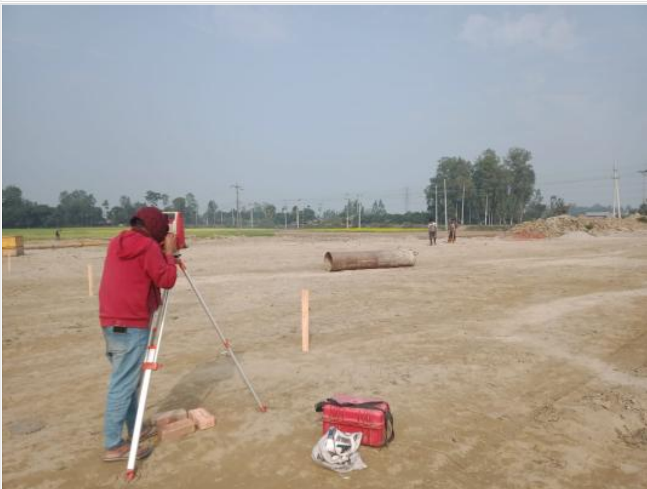
Pile Point Layout and Survey on 01-02-23
