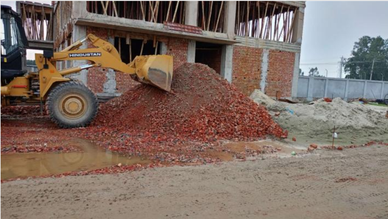
Sub-base-Khoa unloading on 14-08-23
