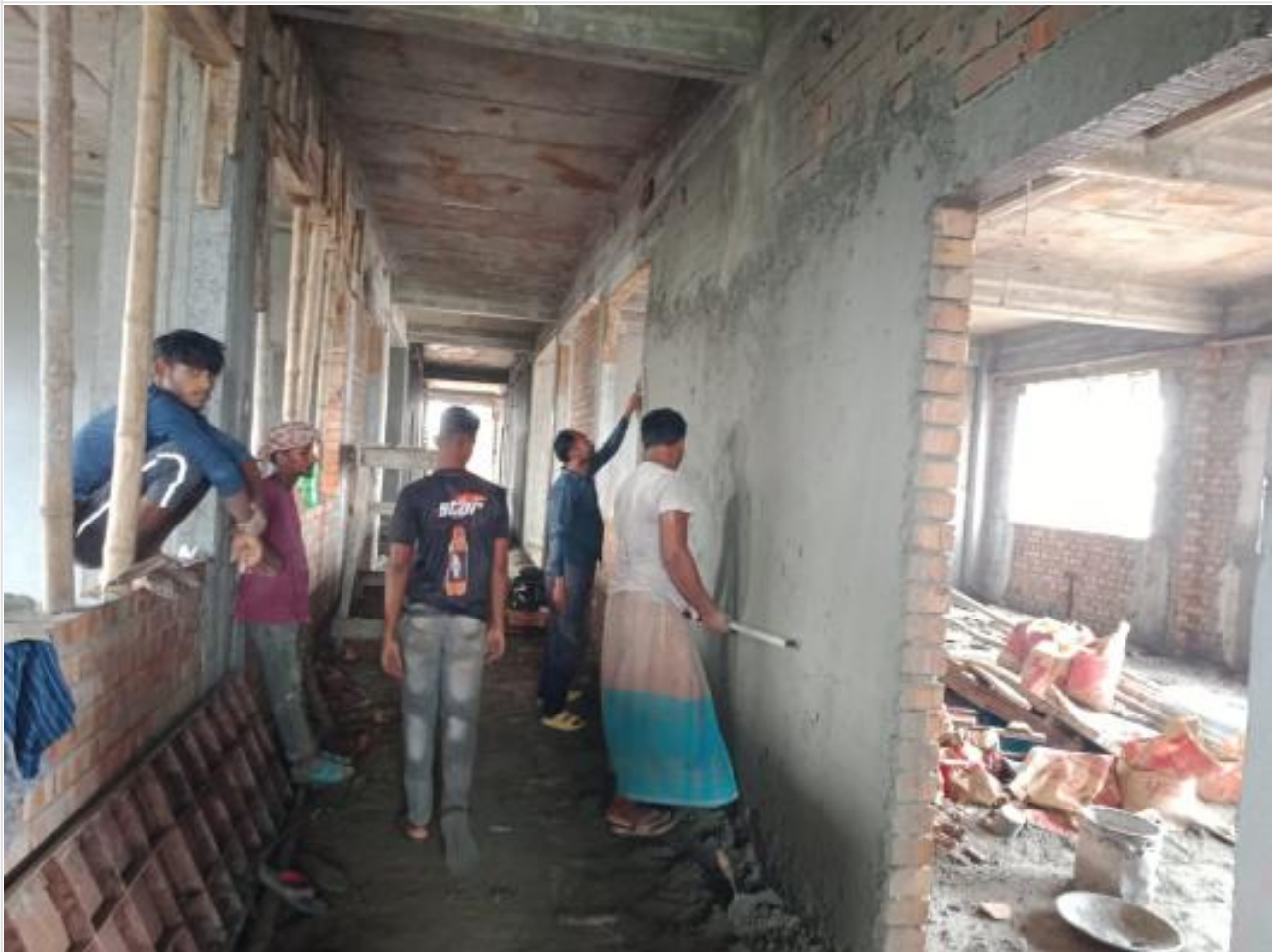
Comp. Bldg. GF plaster work on 27-08-23
