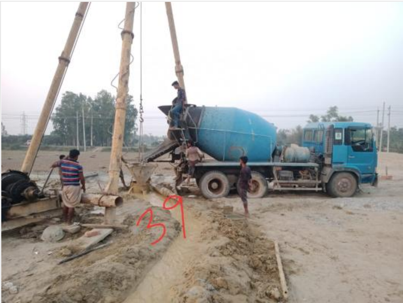
Ready mix concreting of pile on 02-03-23
