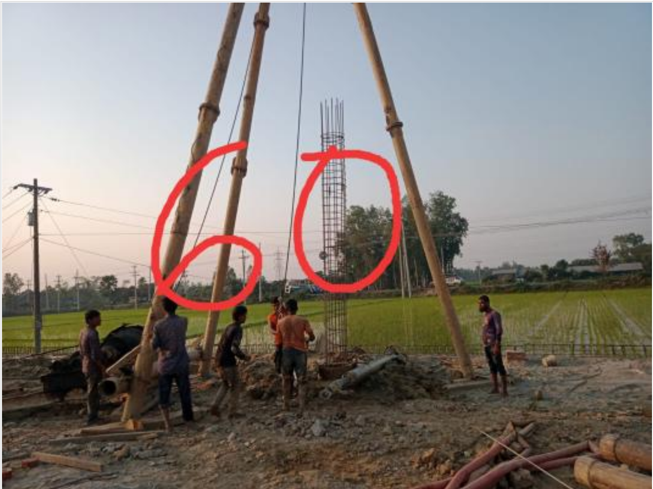
Ready mix concreting of pile on 12-03-23
