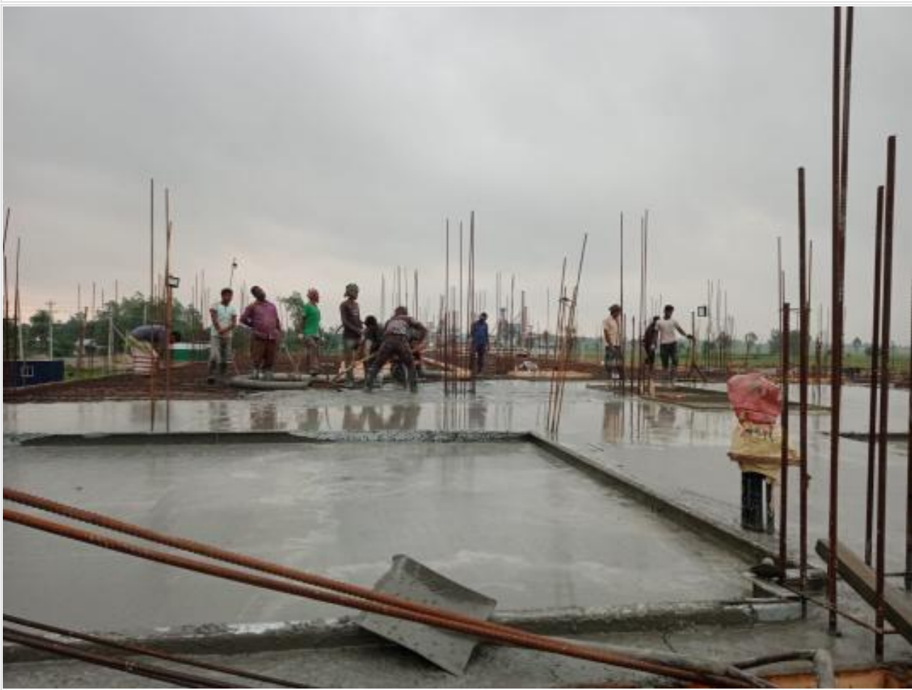
Com. Bldg. 1st floor slab casting on 27-06-23
