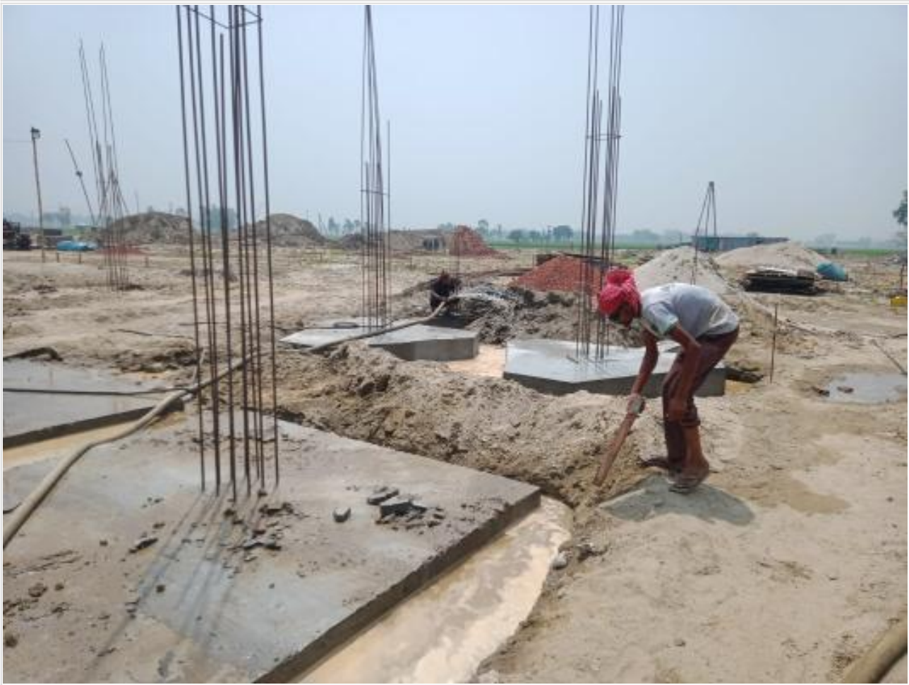
Comp. Bldg. Back filling on 19-04-23
