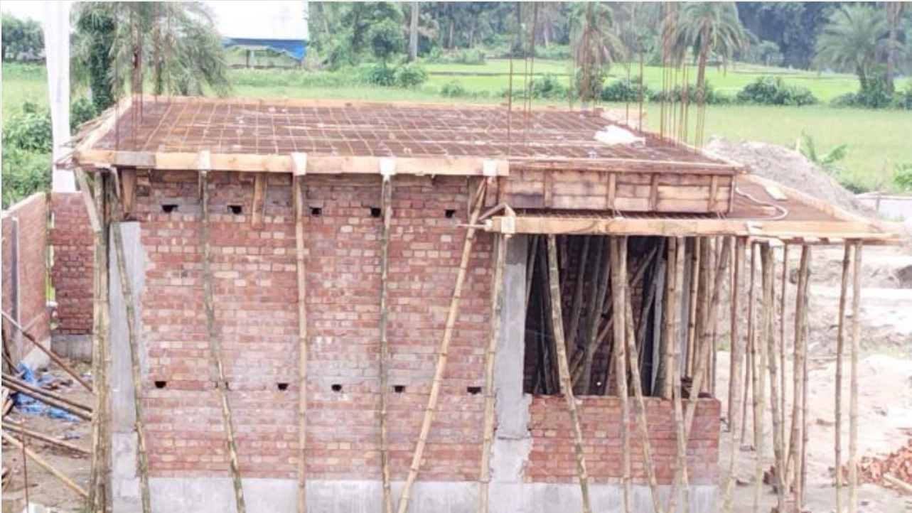
Gate House work on 04-07-23
