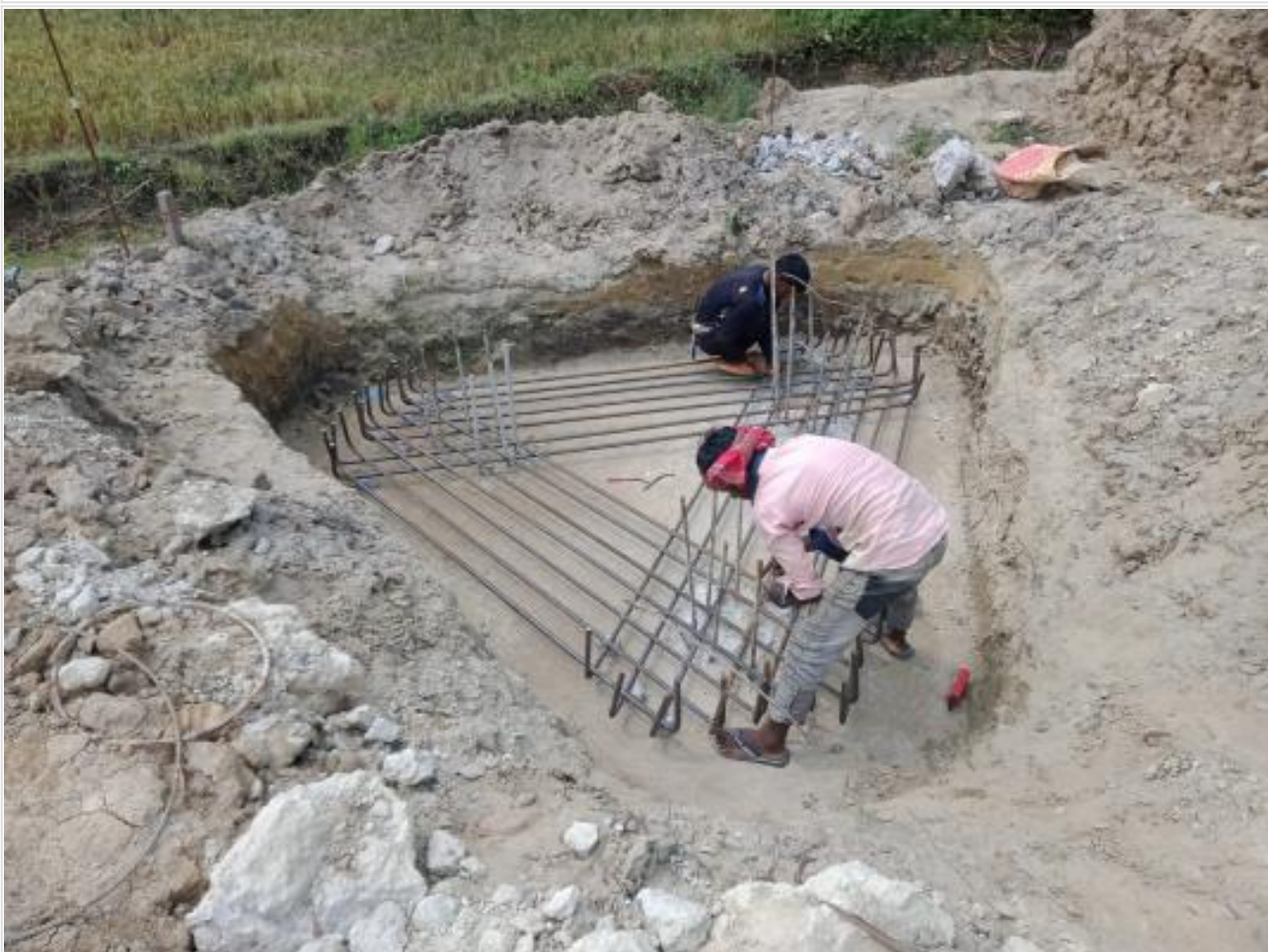
Dorm Bldg pile cap rebar binding on 23-05-23
