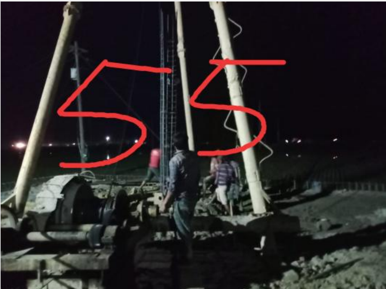
Ready mix concreting of pile on 10-03-23
