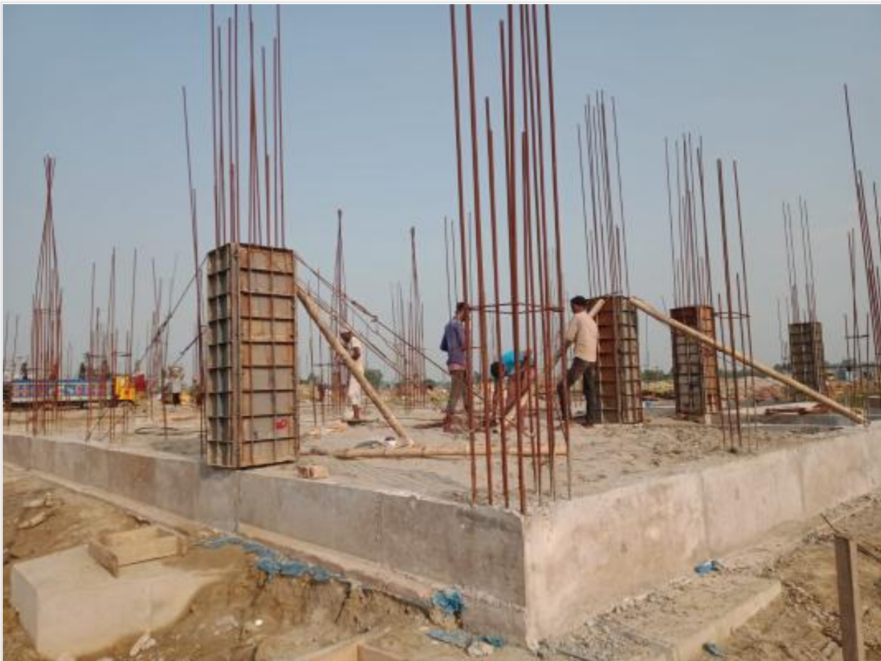
Comp. Bldg. Column shuttering on 24-05-23
