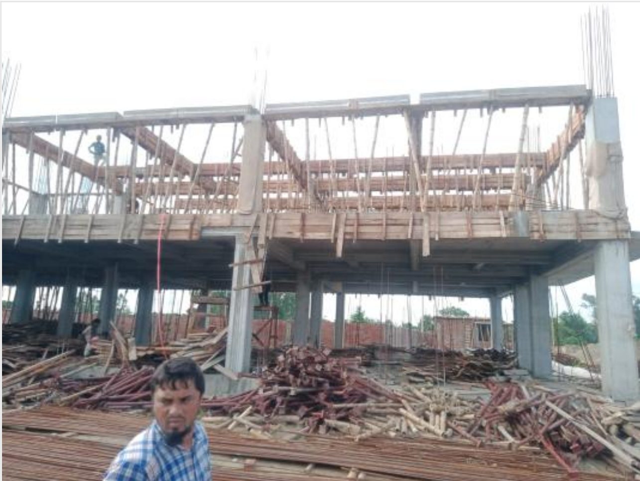
Comp. Bldg. Slab beam shuttering on 17-07-23
