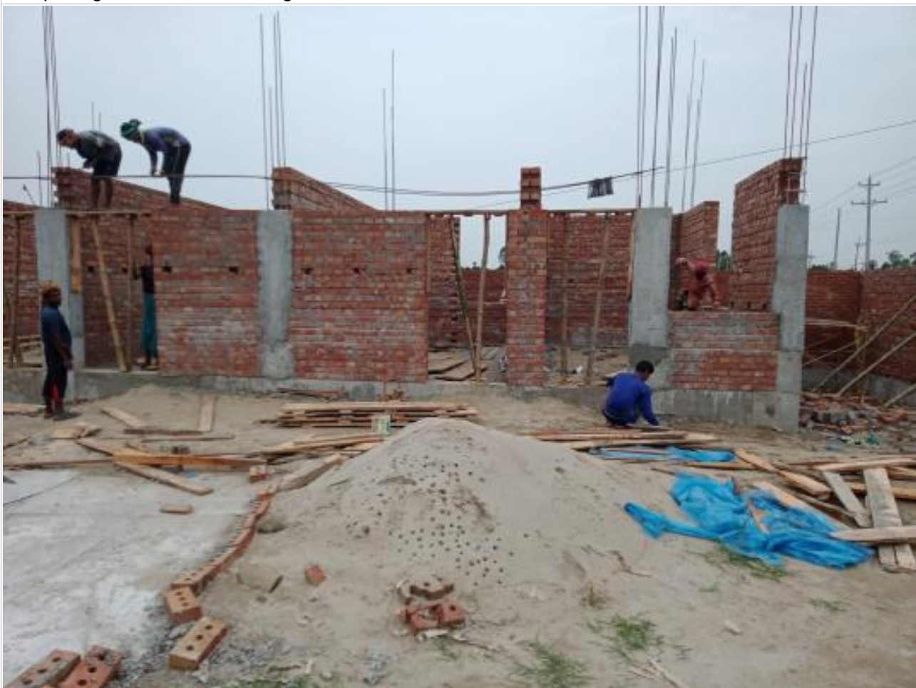
Gate house work on 19-06-23
