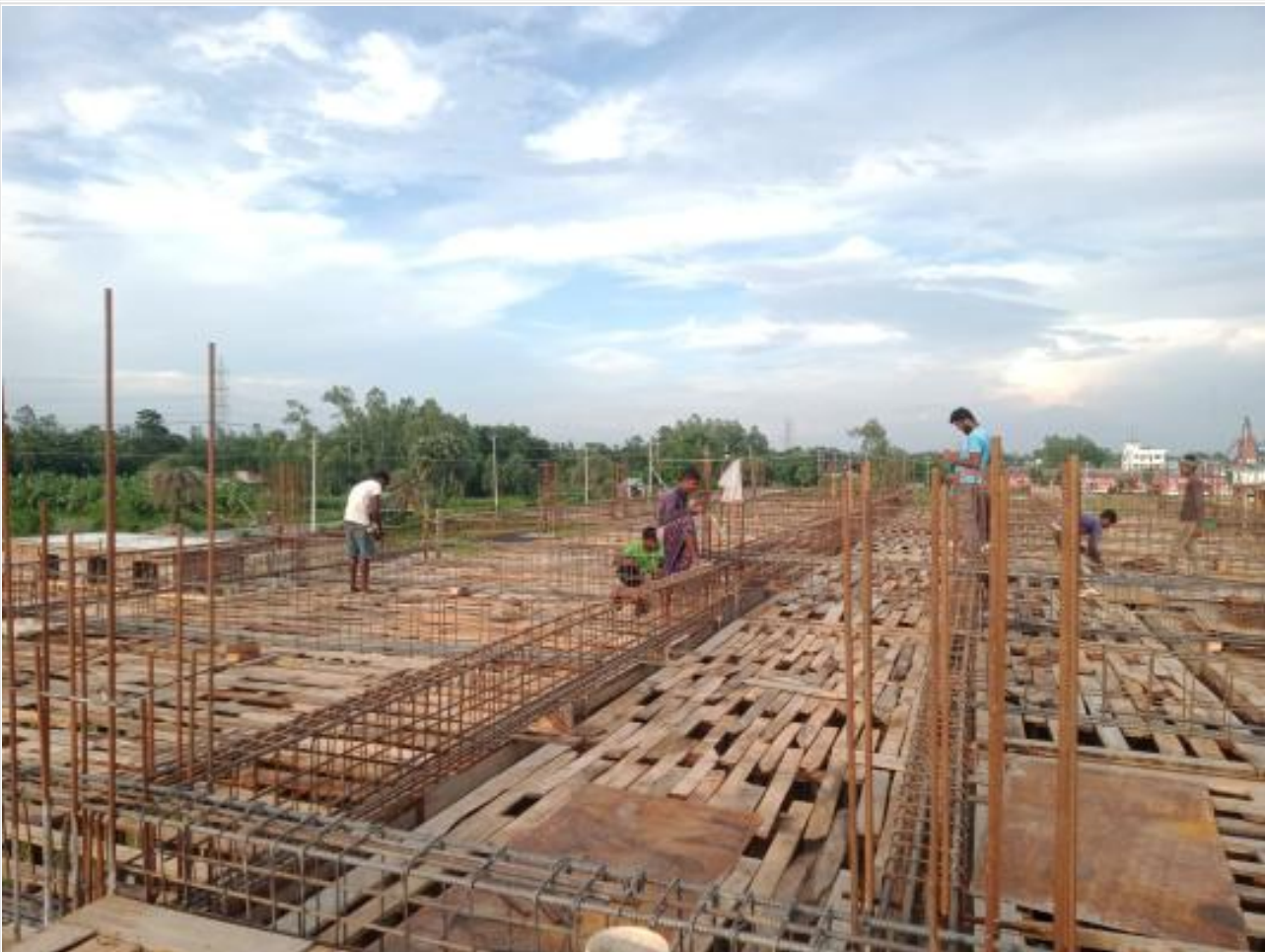
Comp. Bldg. 2nd Floor rebar work on 28-07-23
