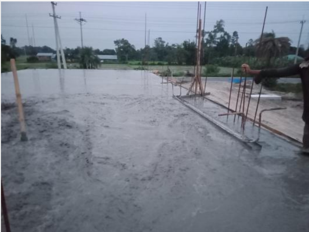
Gate House Slab Casting complete on 11-07-23
