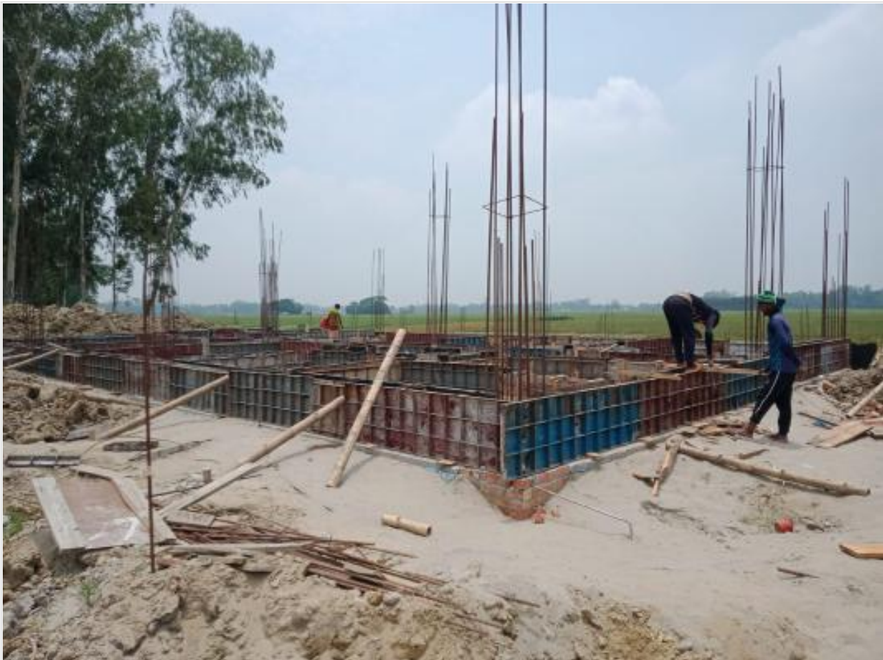
Dorm. Bldg. GB shuttering on 09-06-23
