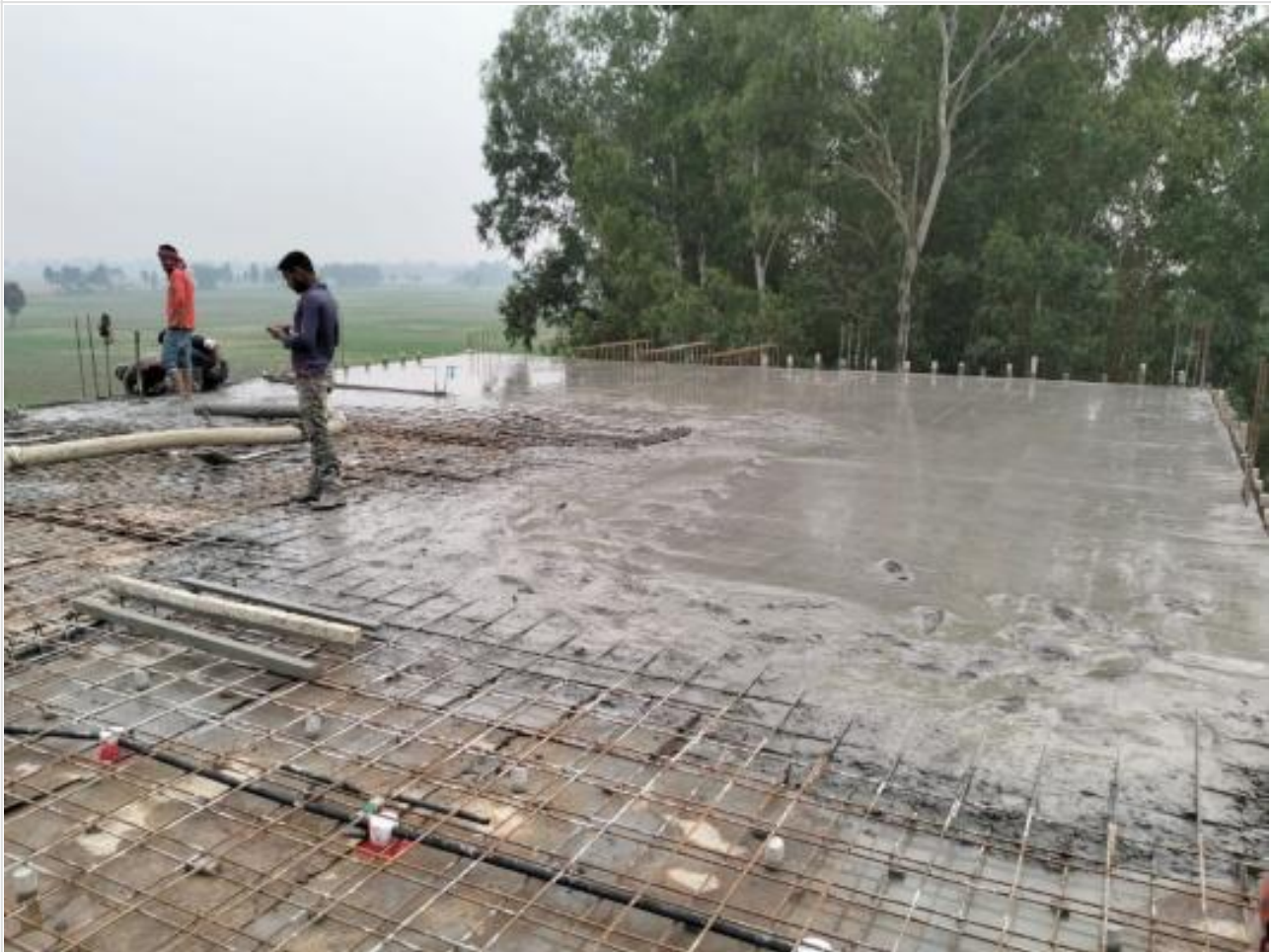
Dormitory-3rd Floor Slab Concreting on 23-12-23
