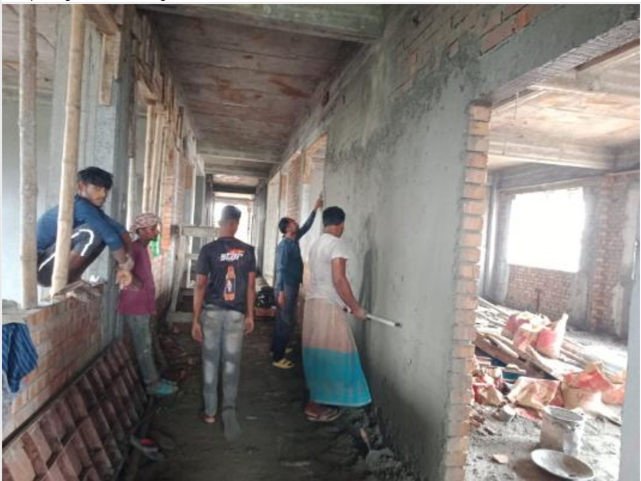
Comp. Bldg. GF plaster work on 27-08-23
