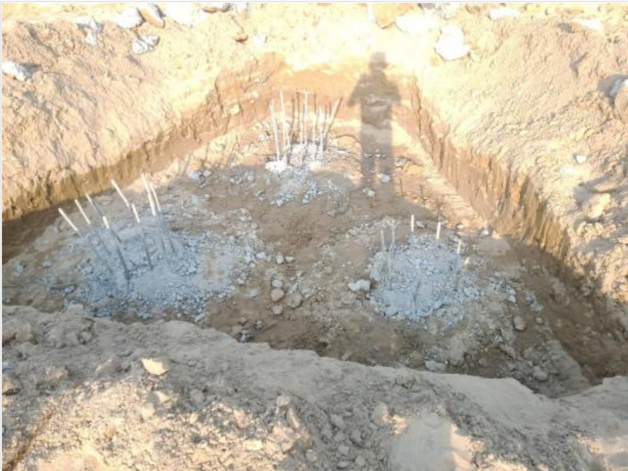
Dorm. Bldg. Pile head breaking on 07-05-23
