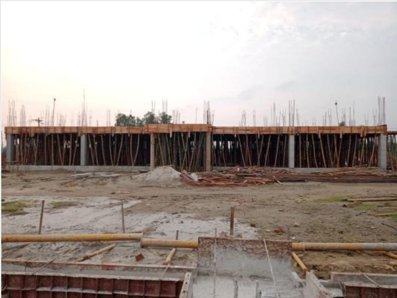
Comp. Bldg. Slab shutter and Rebar work on 22-06-23
