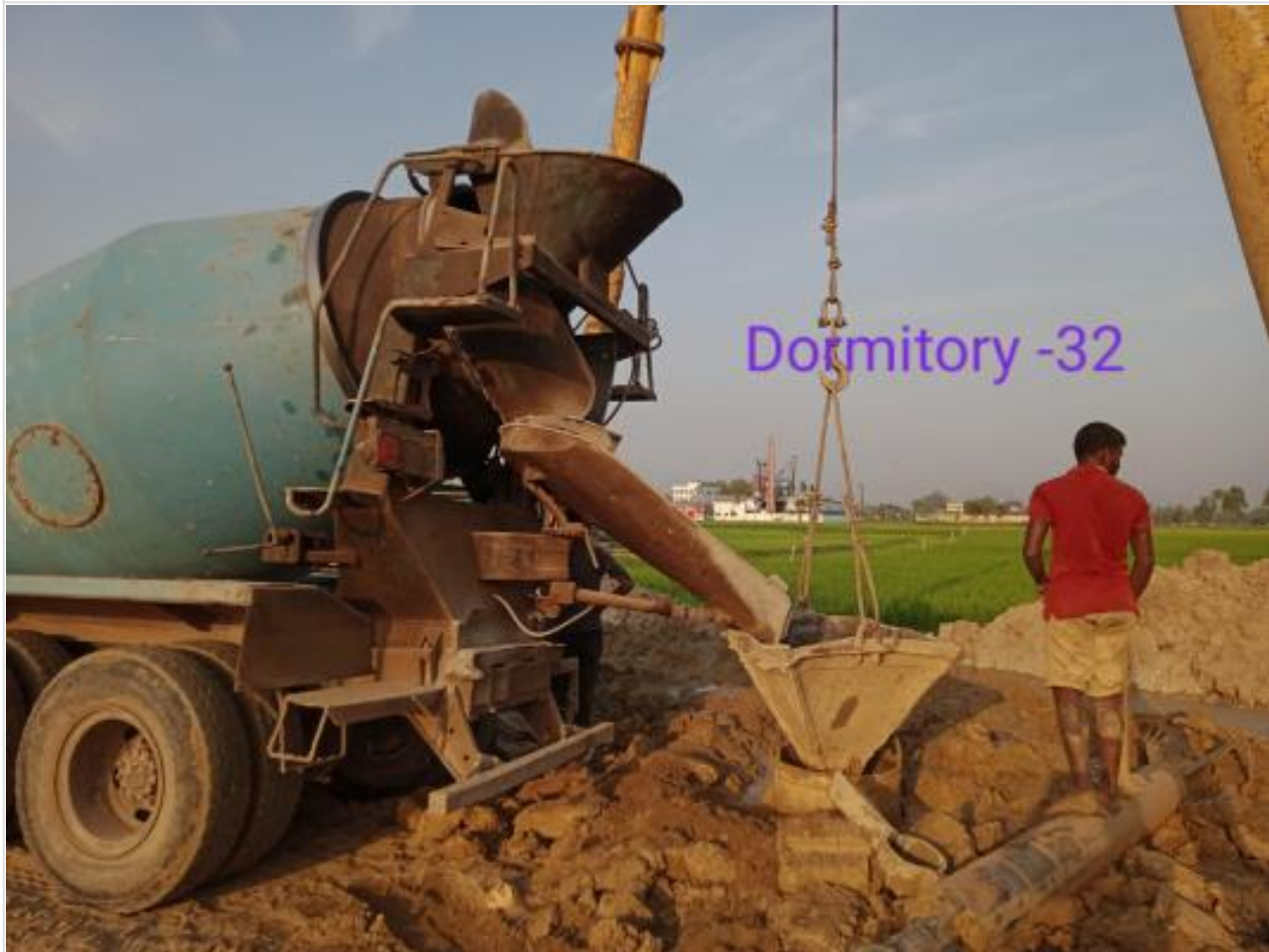
Dorm. Bldg. 32nd pile concreting on 09-04-23
