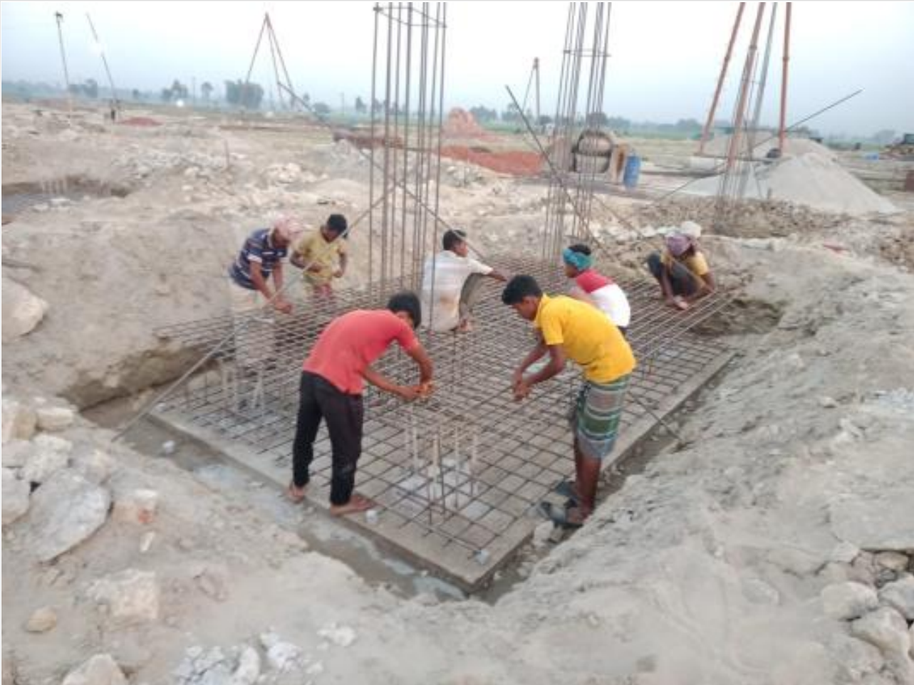
Com. Bldg. Pile cap work on 10-04-23
