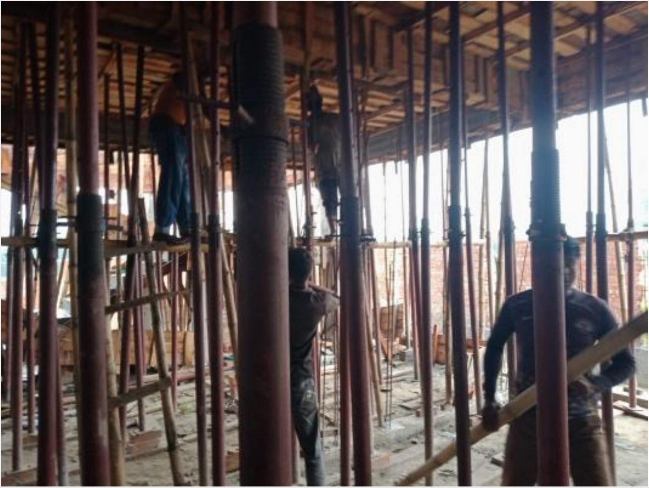
Shuttering work on 09-07-23
