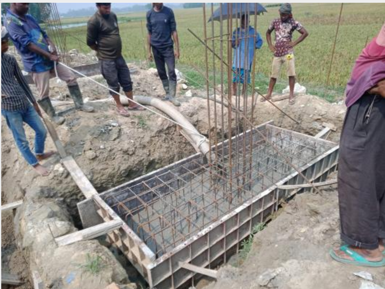
Dorm. Bldg pile cap casting on 28-05-23
