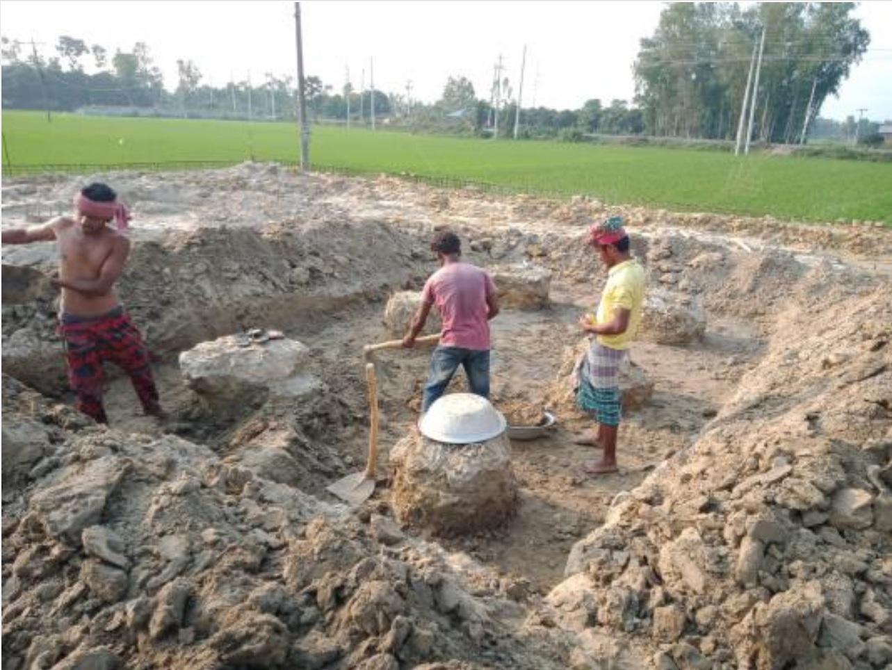
Pile head breaking on 24-03-23
