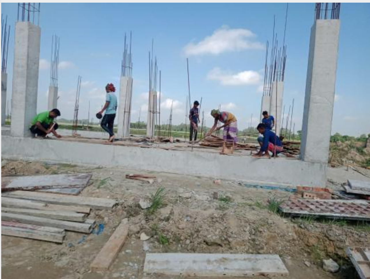
Dorm. Bldg. Floor levelling work on 20-07-23
