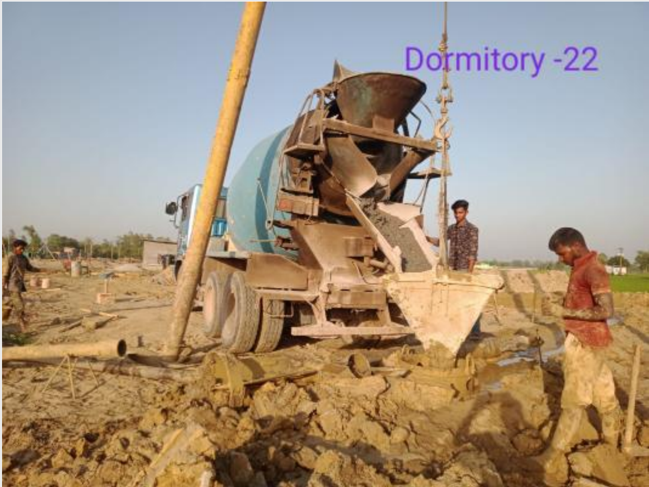
Dorm. Bldg. 22nd pile casting on 06-04-23
