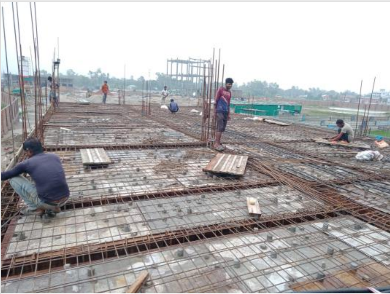
Dormitory Slab Electric Pipe Laying on 09-08-23
