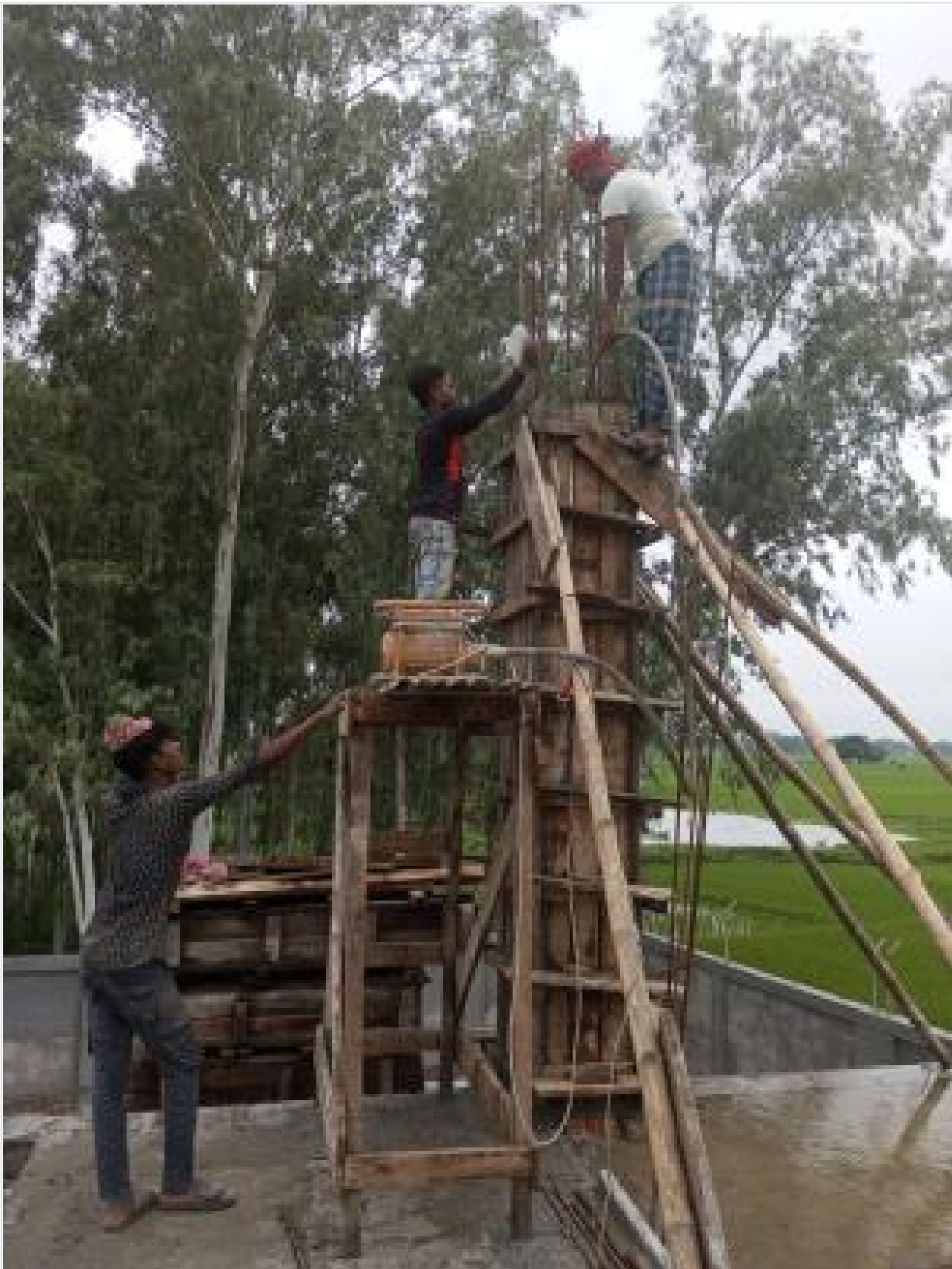
Column casting work on 25-08-23
