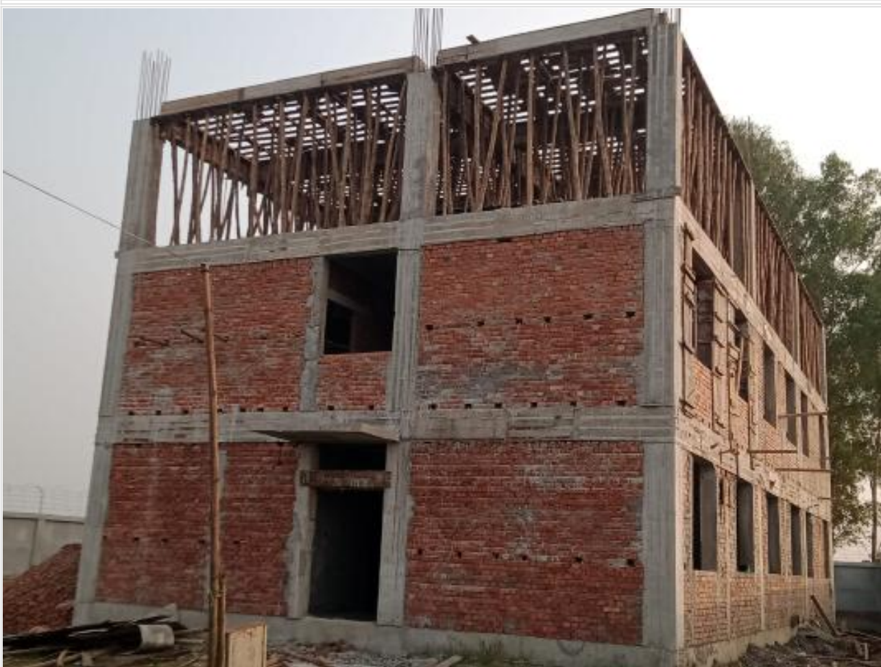
Dorm. Bldg. 3rd floor shuttering work on 09-11-23
