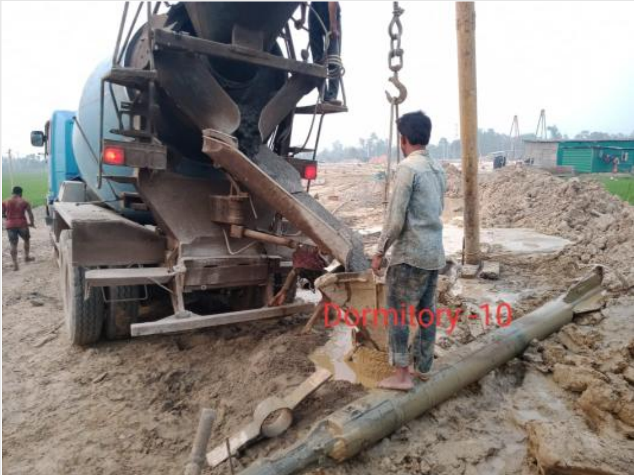
Dorm. Bldg. 10th pile concreting on 30-03-23
