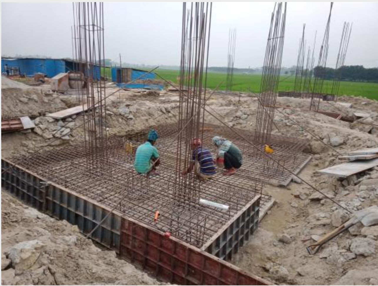
Pile Cap rebar binding on 15-04-23
