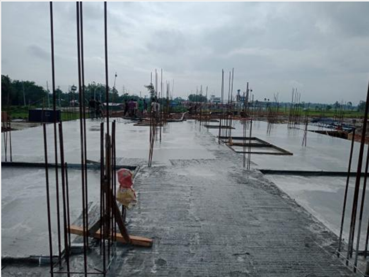
Comp. Bldg. Slab casting complete on 27-06-23
