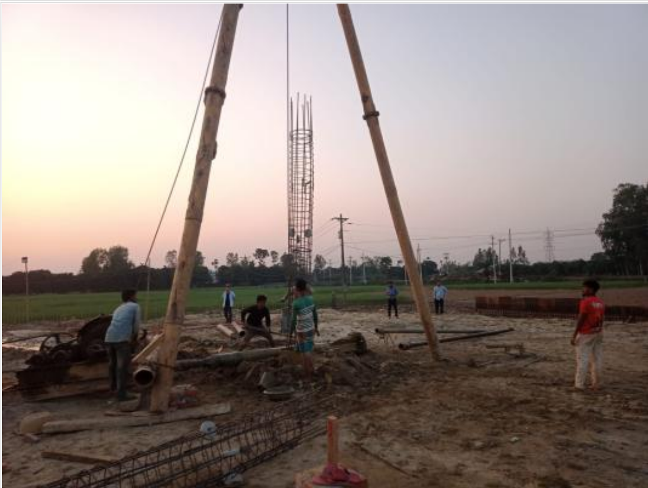
Pile boring work on 14-02-23
