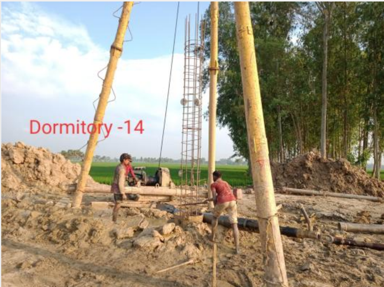
Ready mix concreting of pile on 31-03-23
