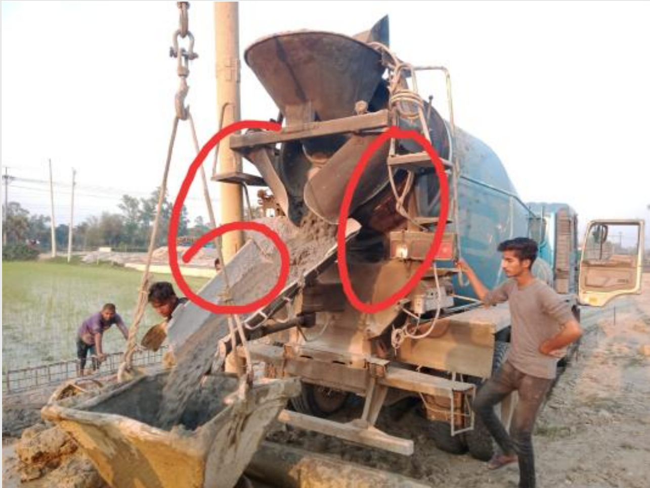
Ready mix concreting of pile on 13-03-23
