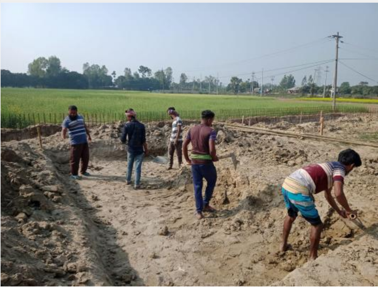
Exaction for Pile mud tank on 02-02-23
