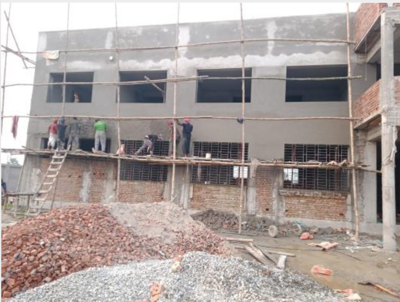
Comp. Bldg. Outside plaster work on 16-10-23
