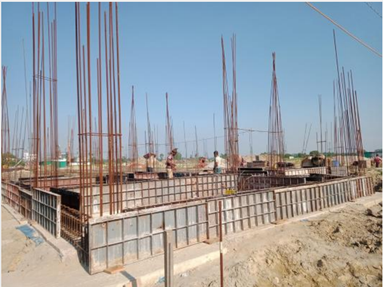
Comp. GB Shuttering on 06-05-23
