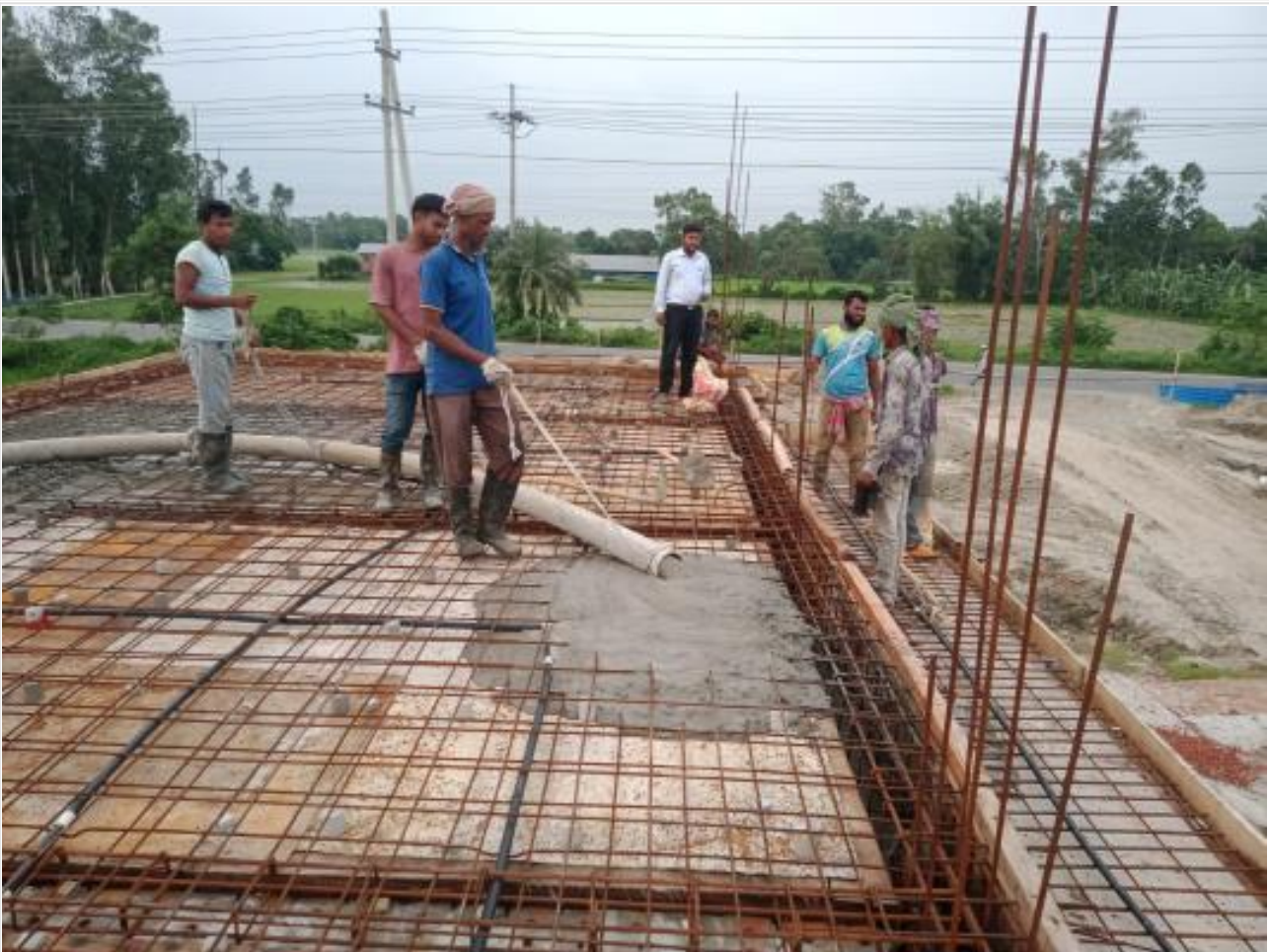
Gate House Slab casting on 11-07-23
