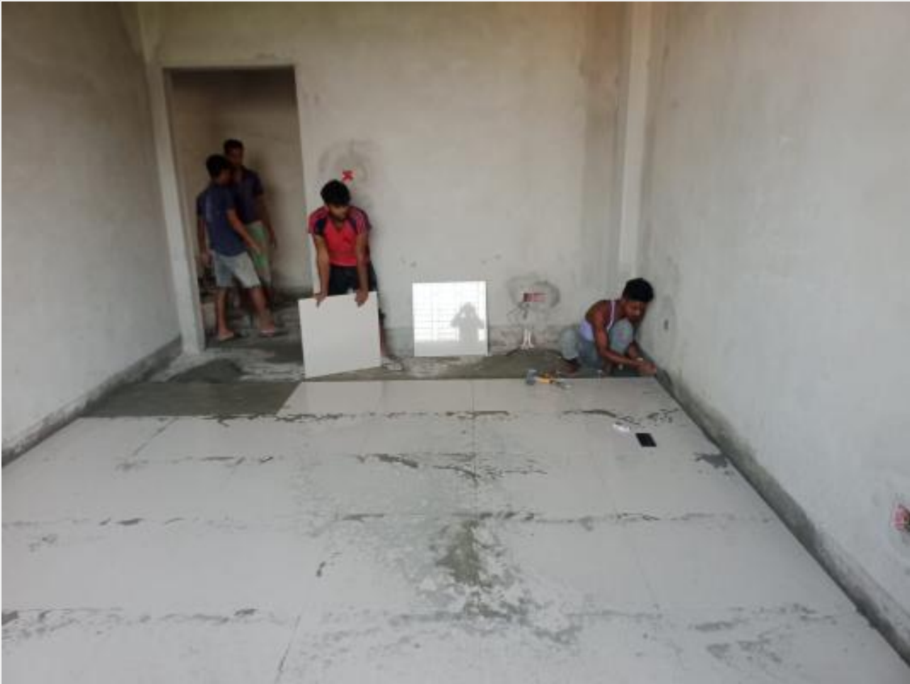
Comp. Bldg. GF Tiles work on 01-11-23
