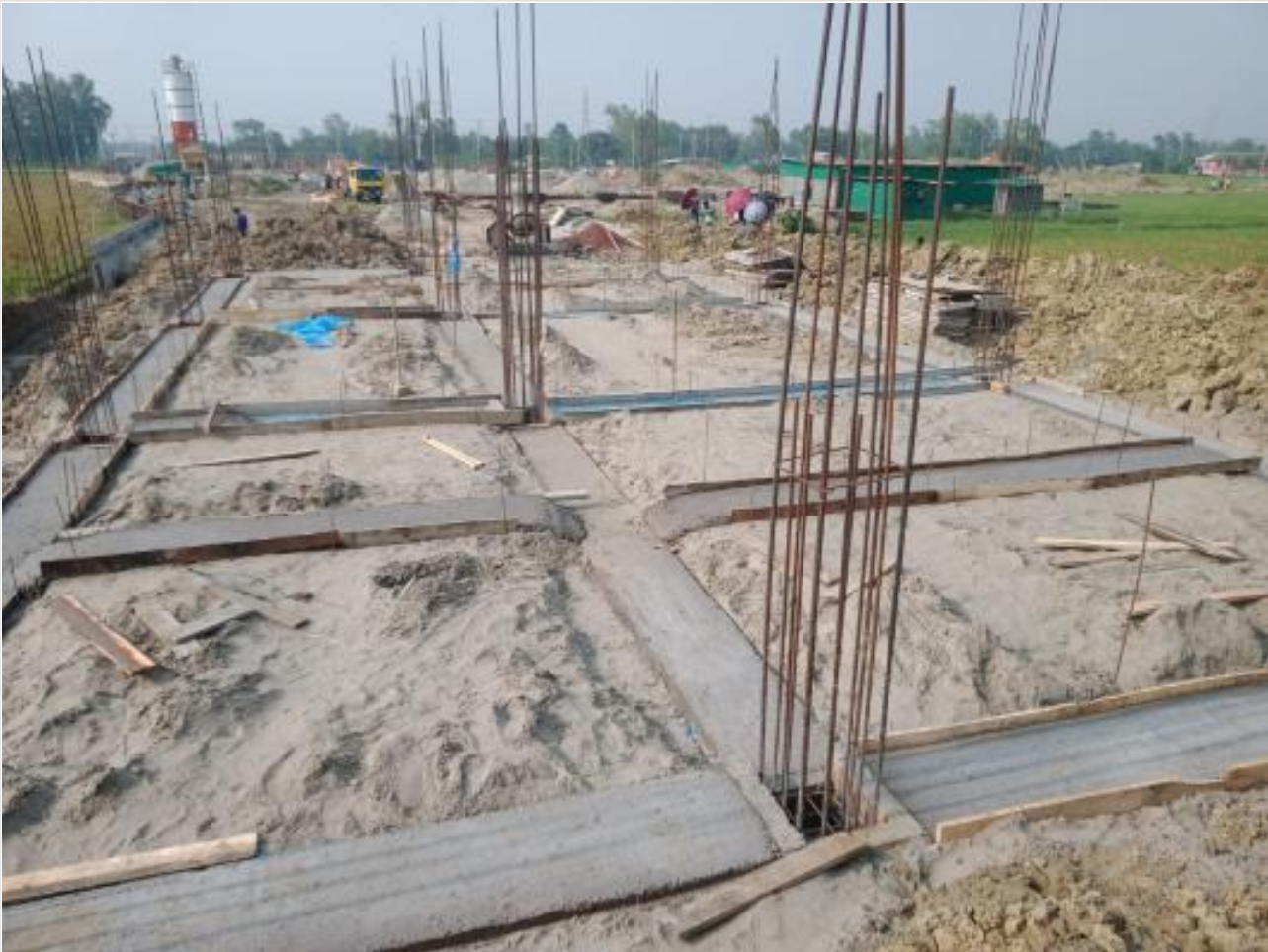
Dorm. Bldg. GB Bottom CC work on 03-06-23
