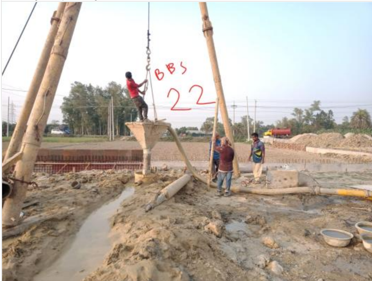
Ready mix concreting of pile on 23-02-23
