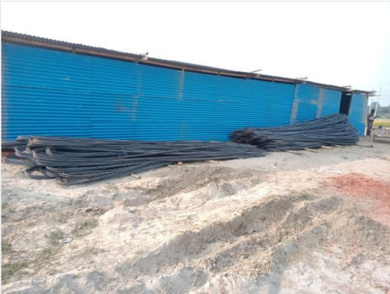
Shed completed on 22-01-23
