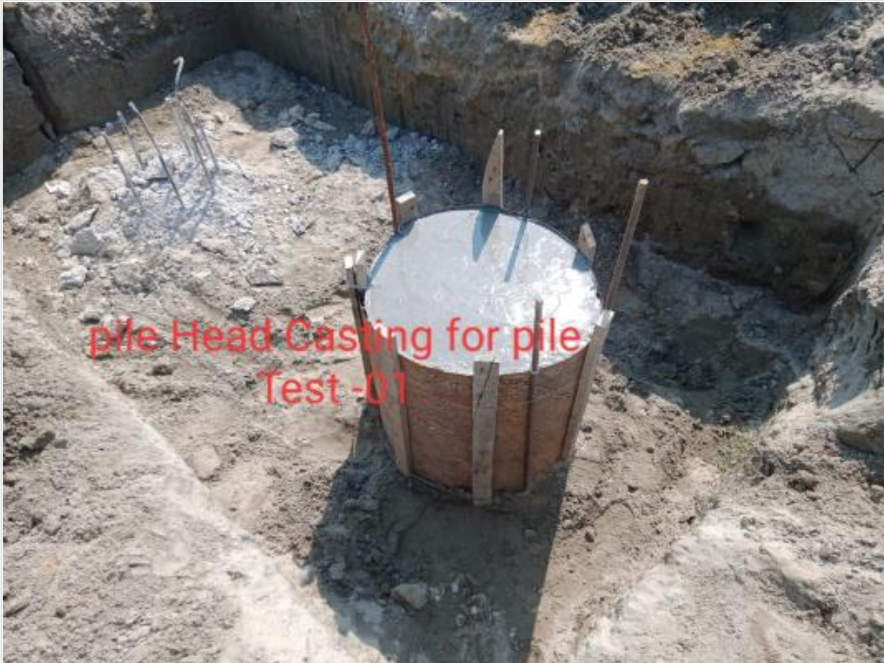
Pile head finishing for test on 03-04-23
