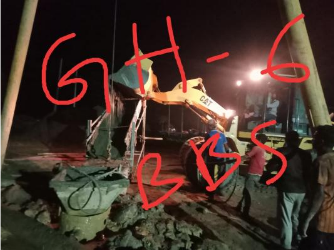
Ready mix concreting of pile on 21-03-23
