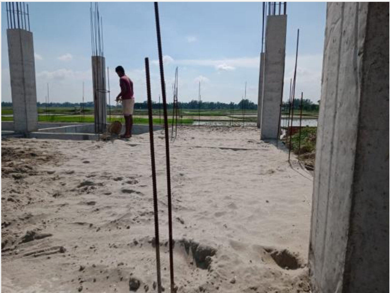
Dorm. Bldg. Sand filling on 18-07-23
