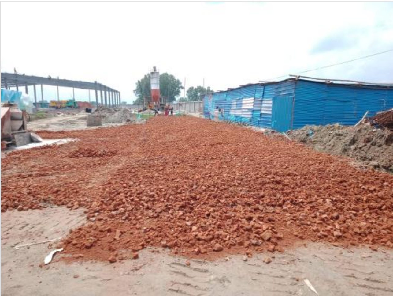
Road Sub-base work on 08-09-23
