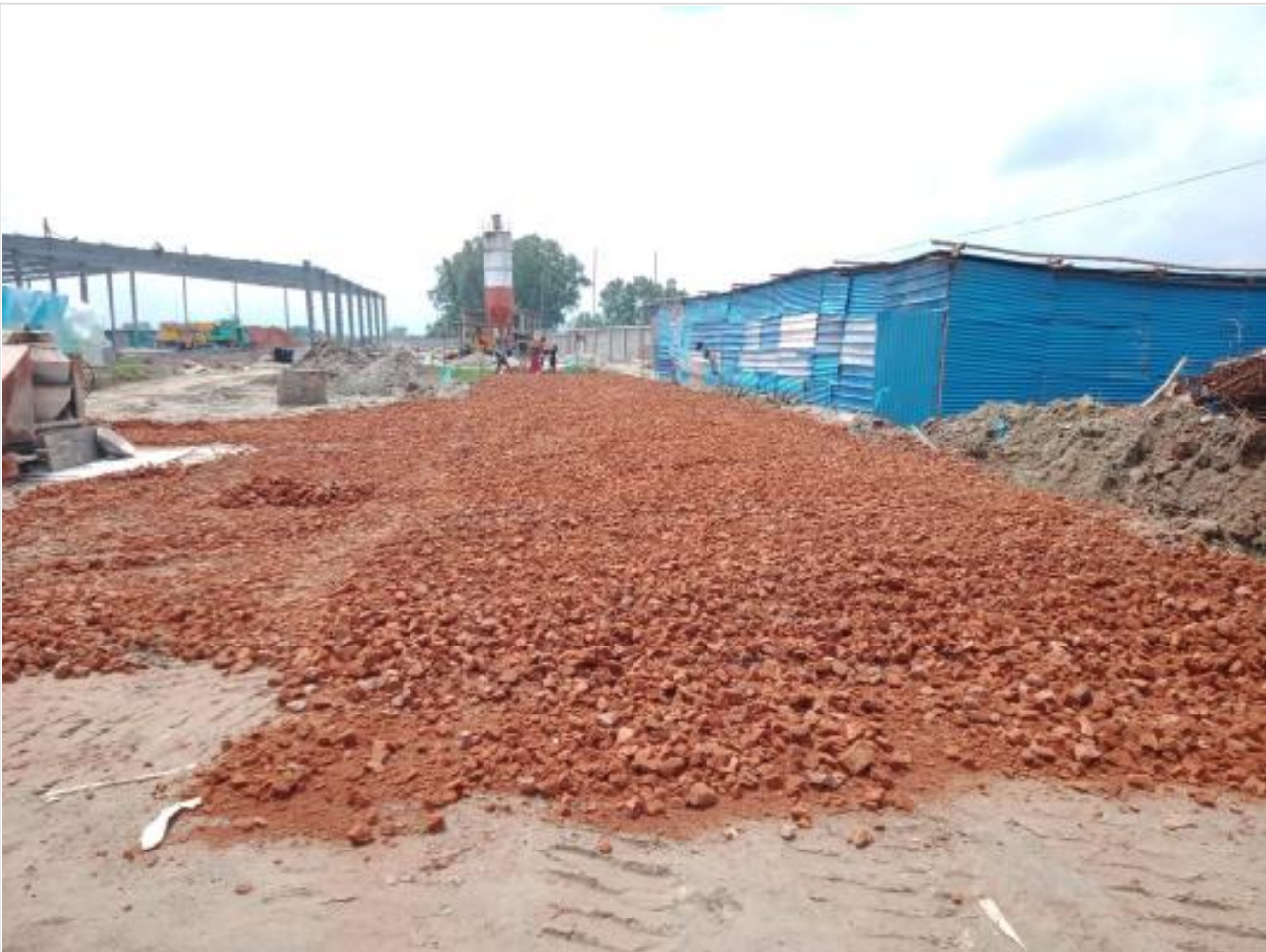
Road Sub-base work on 08-09-23
