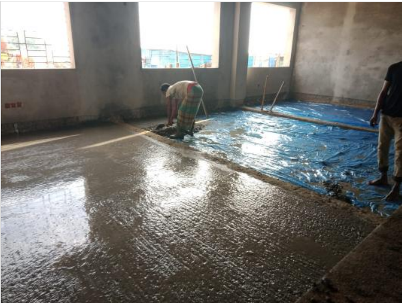
Comp. GF concreting on 29-09-23
