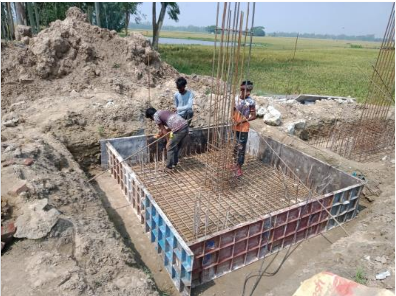
Dorm. Bldg pile cap work on 25-05-23
