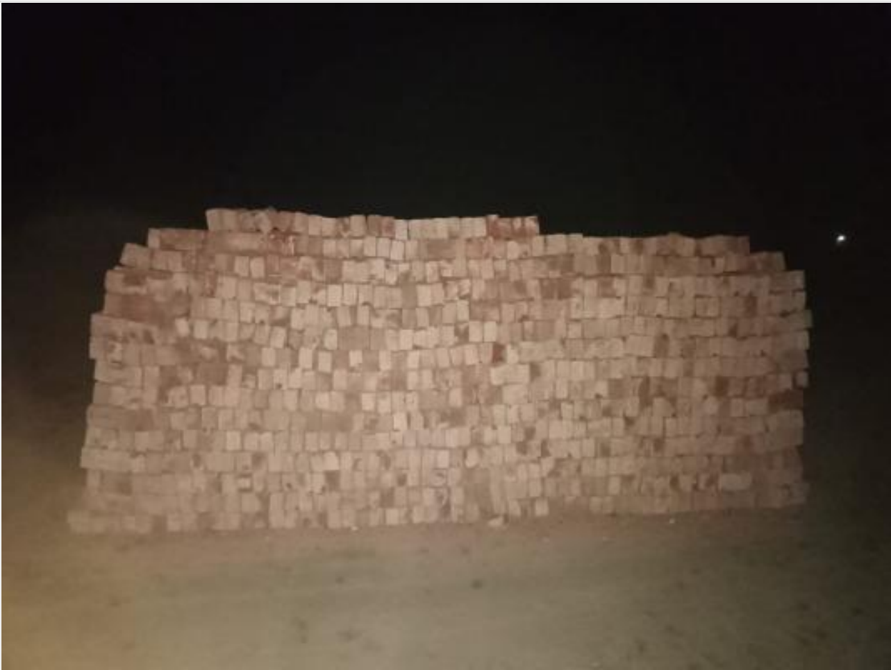
Brick mobilized for shed on 09-01-23
