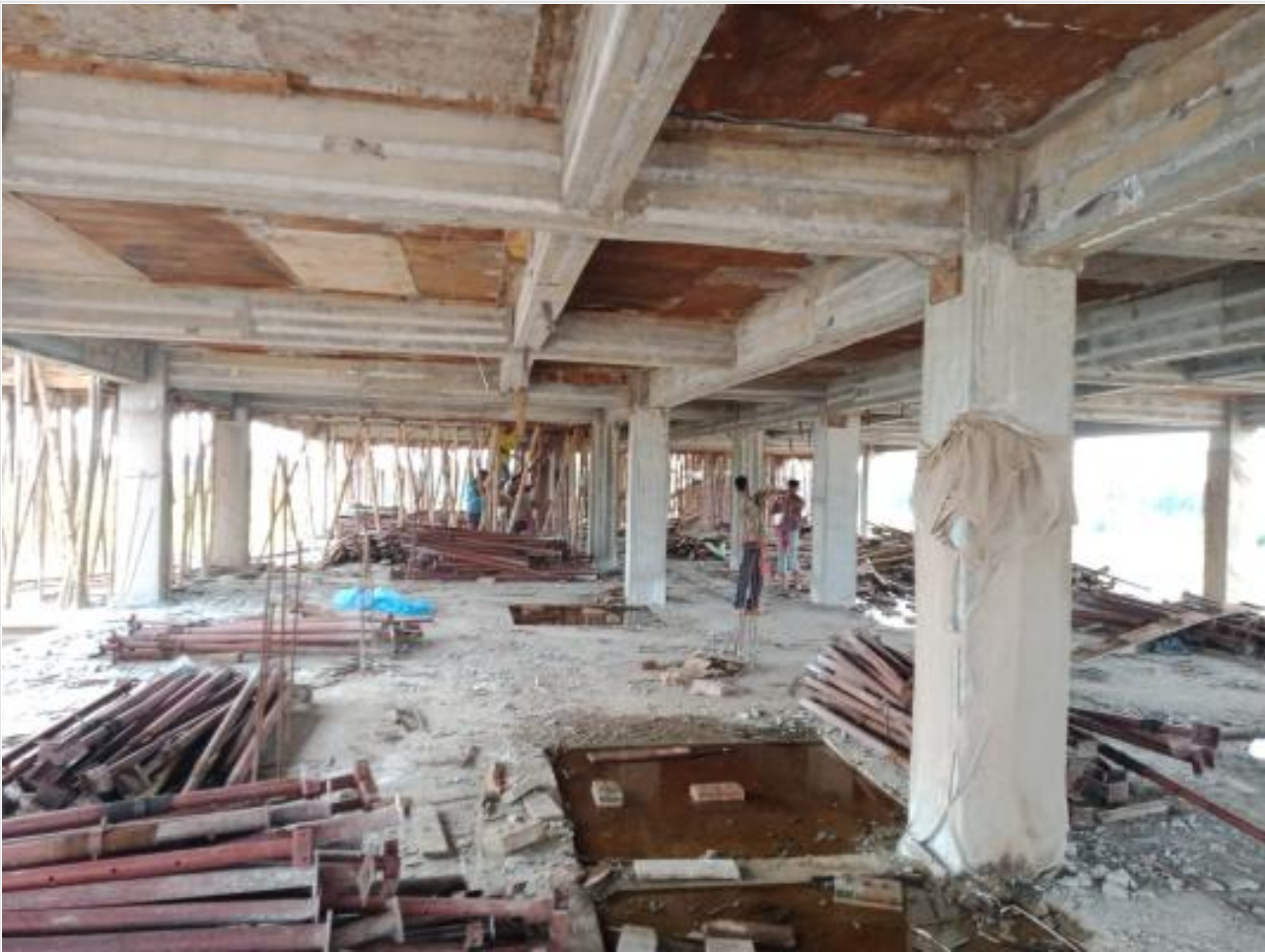
Comp-1st Floor-Shutter Removing on 20-08-23
