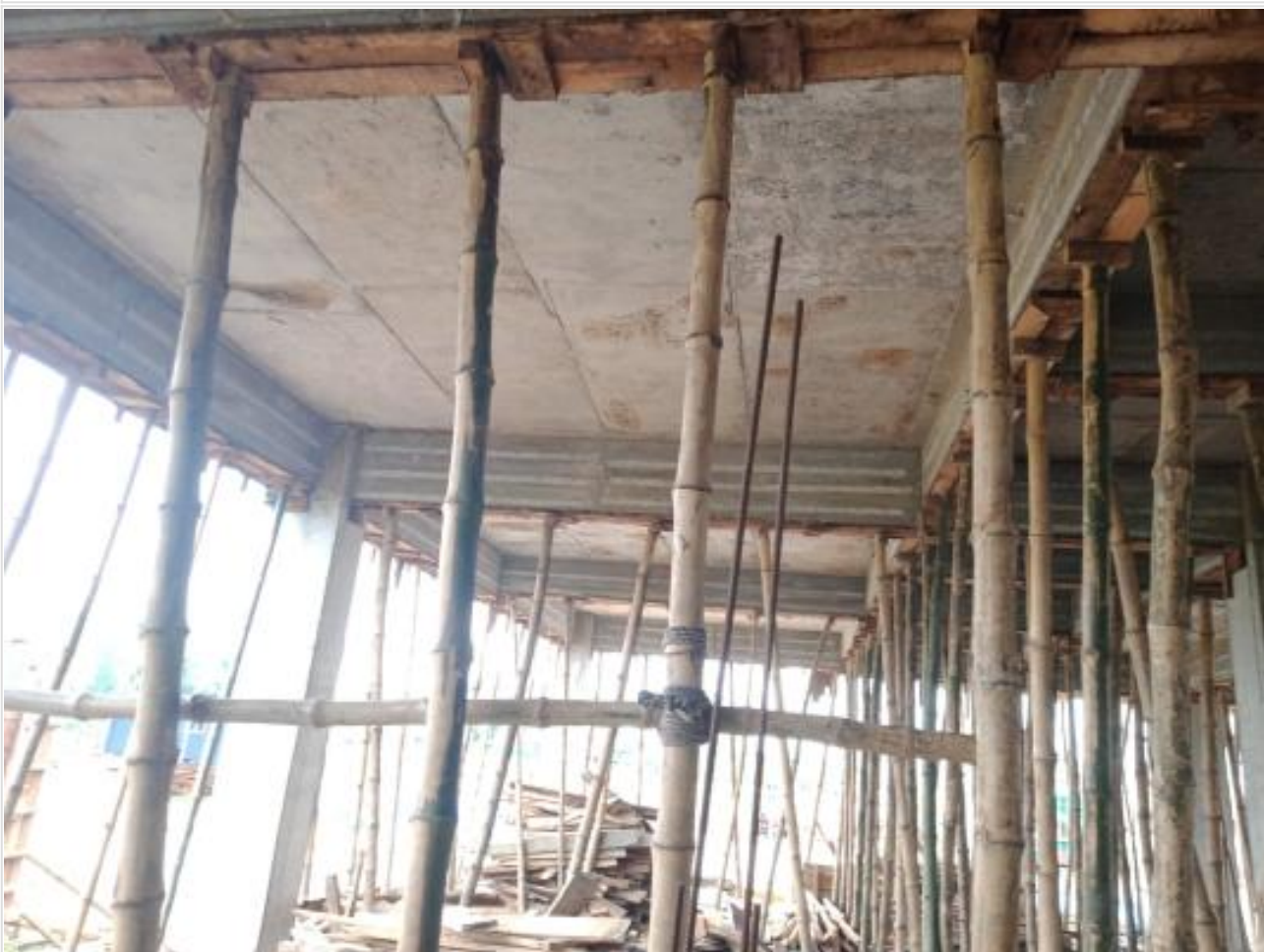
Comp. Bldg. Slab shutter opening on 12-07-23
