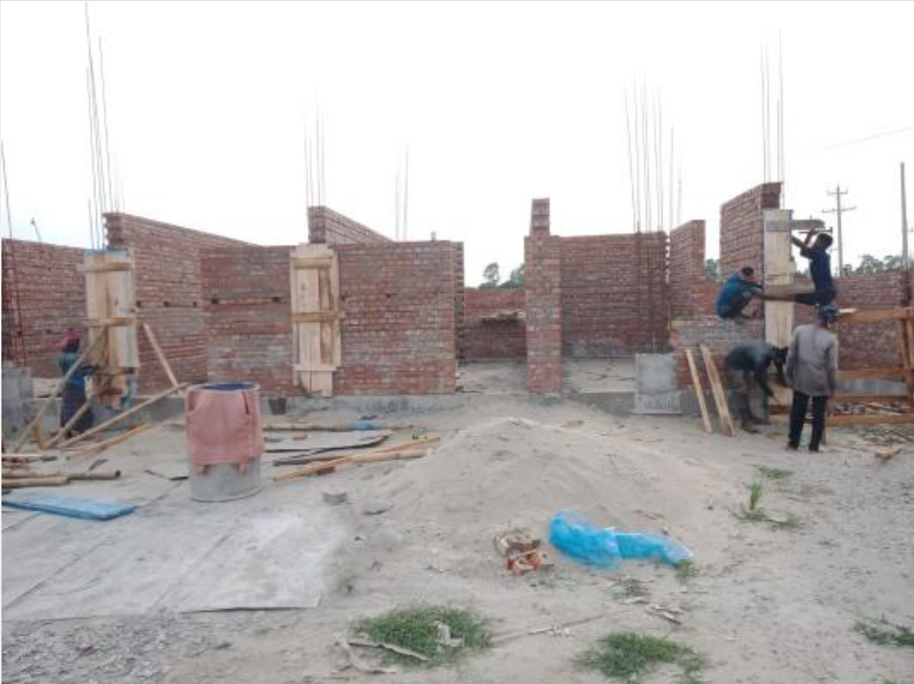
Gate house column shuttering work on 16-06-23
