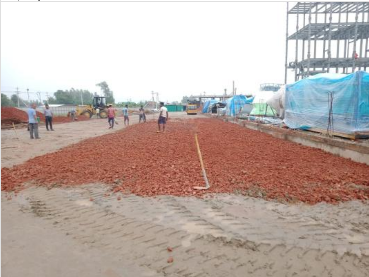
Road work on 24-08-23
