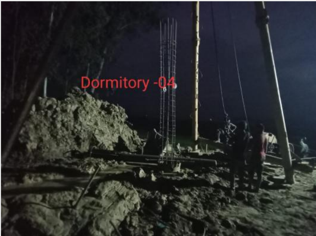
Ready mix concreting of pile on 25-03-23
