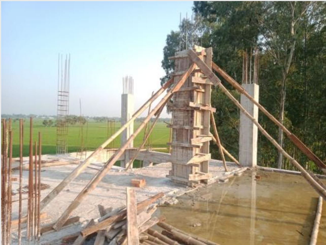
Dorm. Bldg. Roof top Column work on 13-10-23
