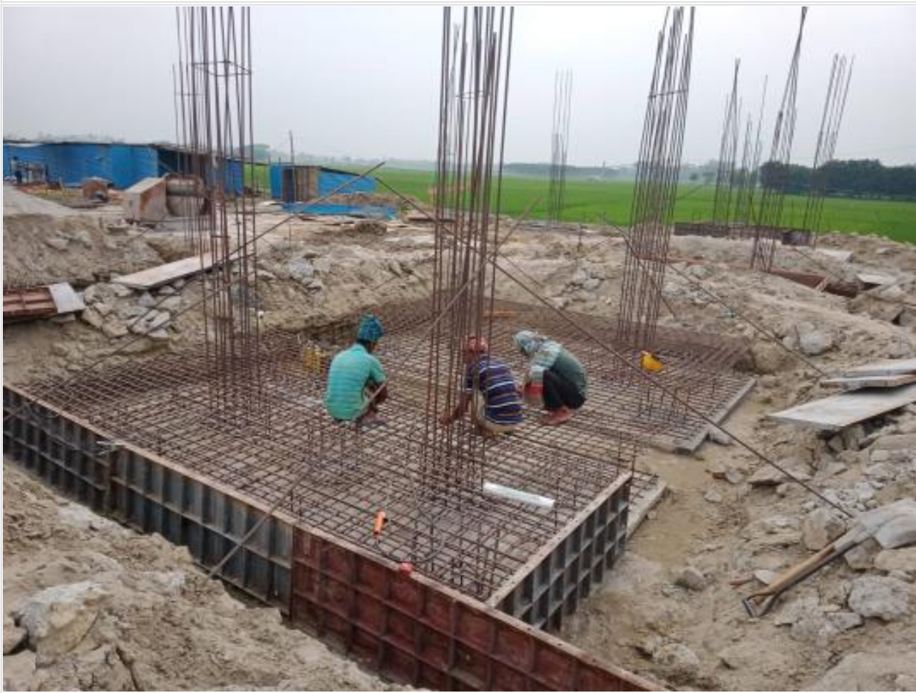
Pile Cap rebar binding on 15-04-23
