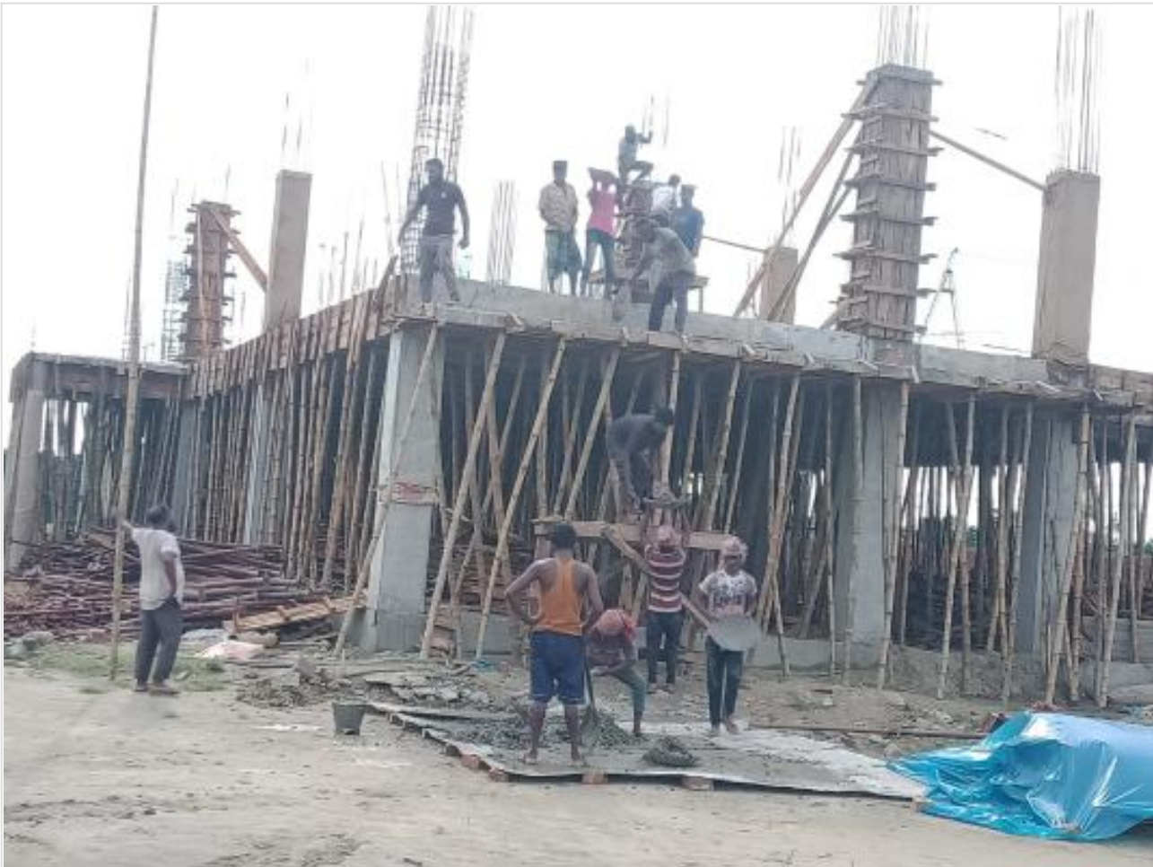
Comp. Bldg. 1st floor column casting on 12-07-23
