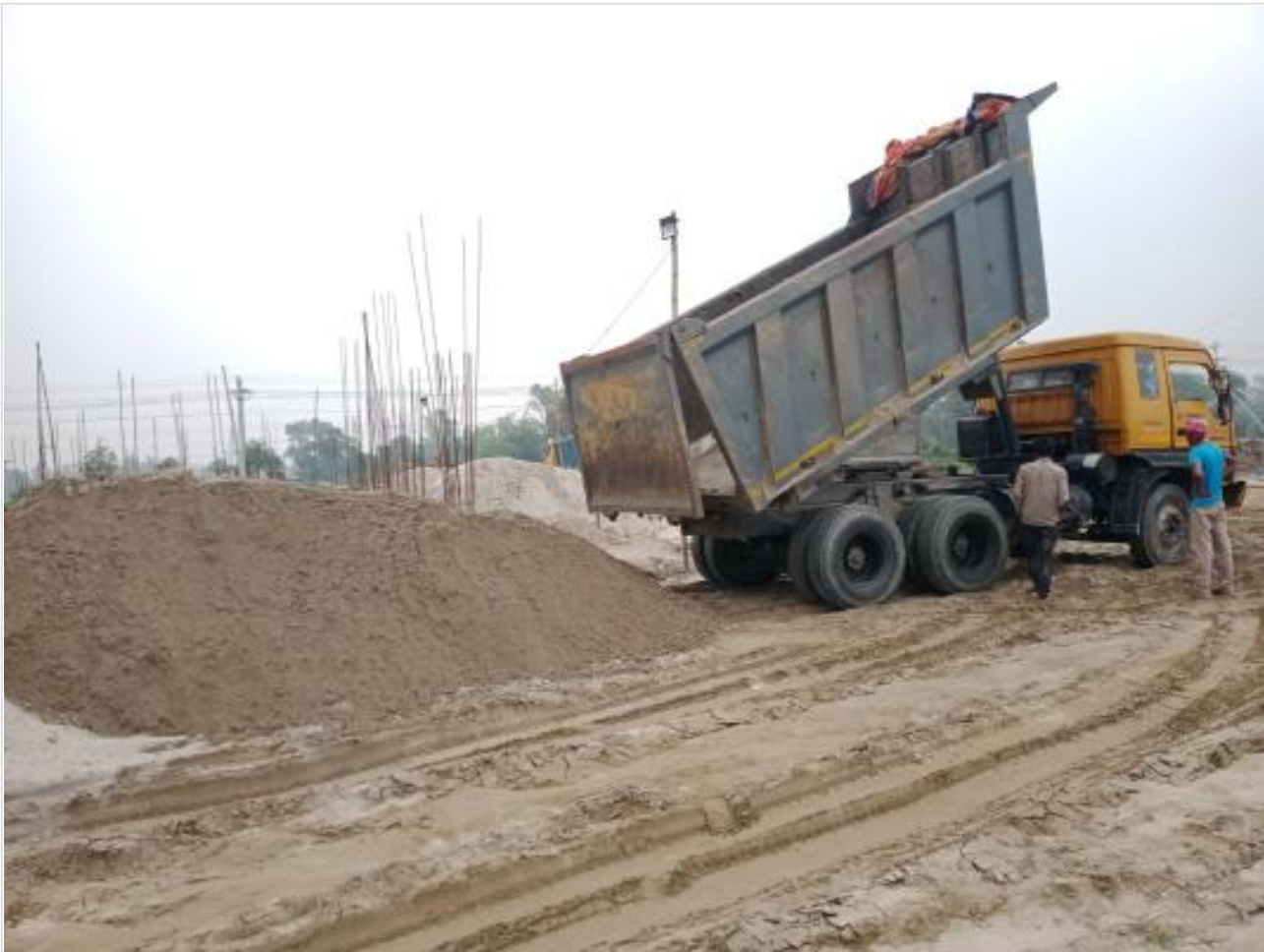
Sand filling on 21-05-23
