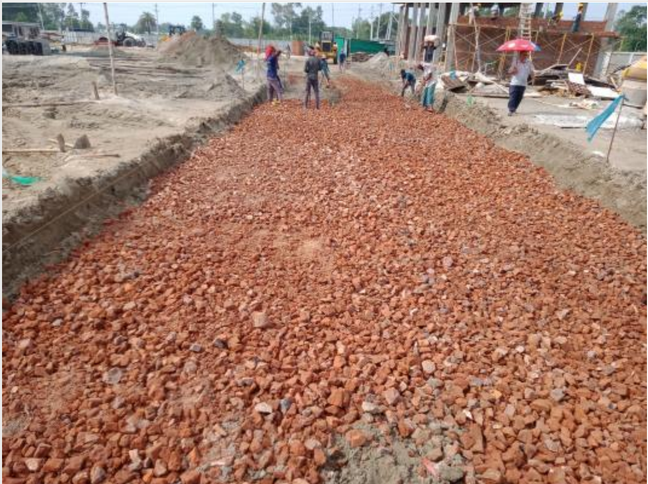
Road-Sub-base work on 21-08-23
