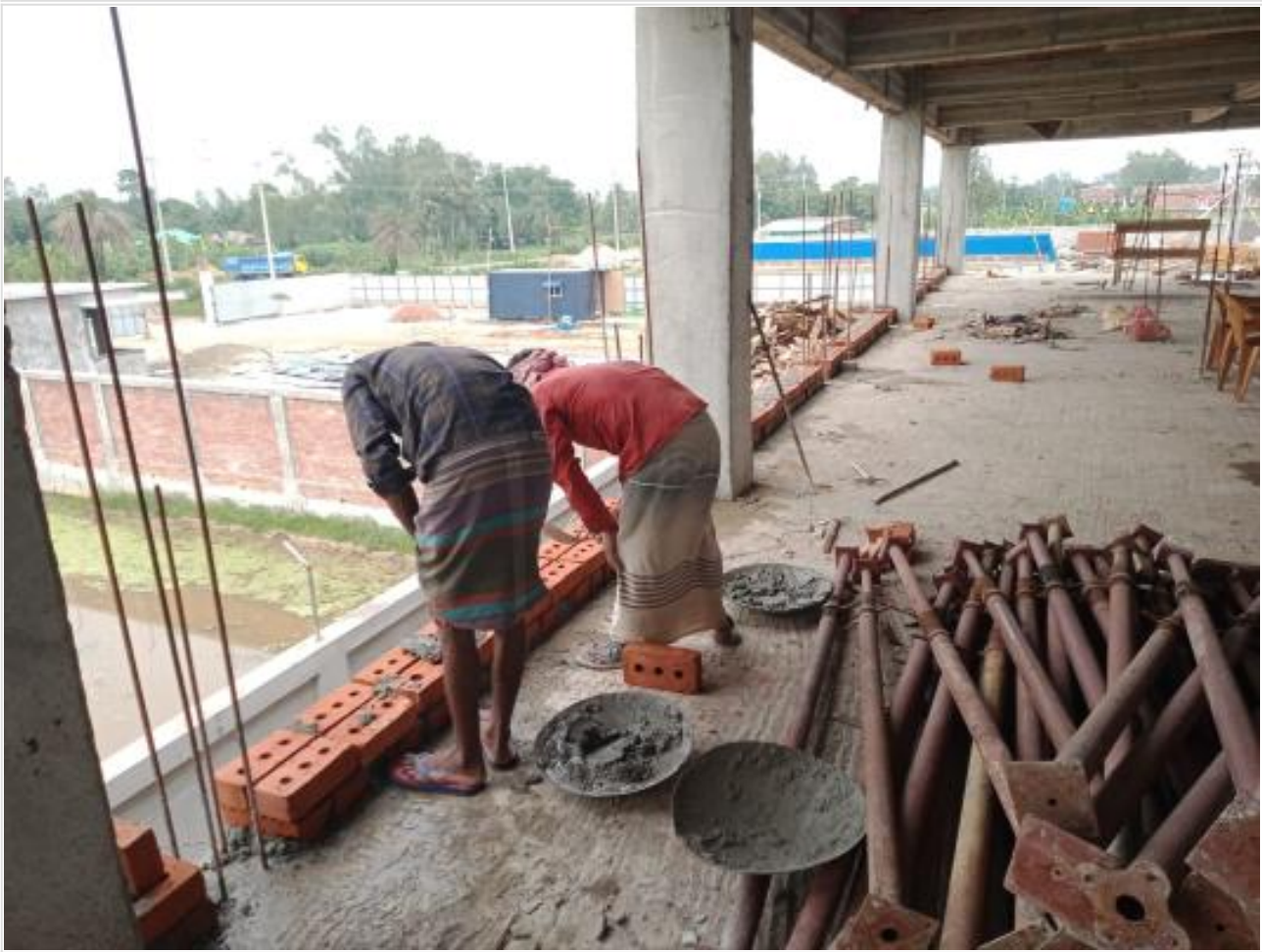
Comp-1st Floor-Brickwork on 22-08-23
