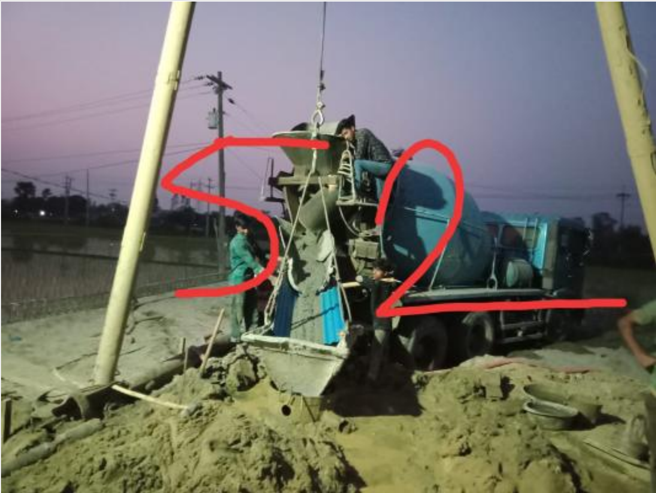
Ready mix concreting of pile on 10-03-23
