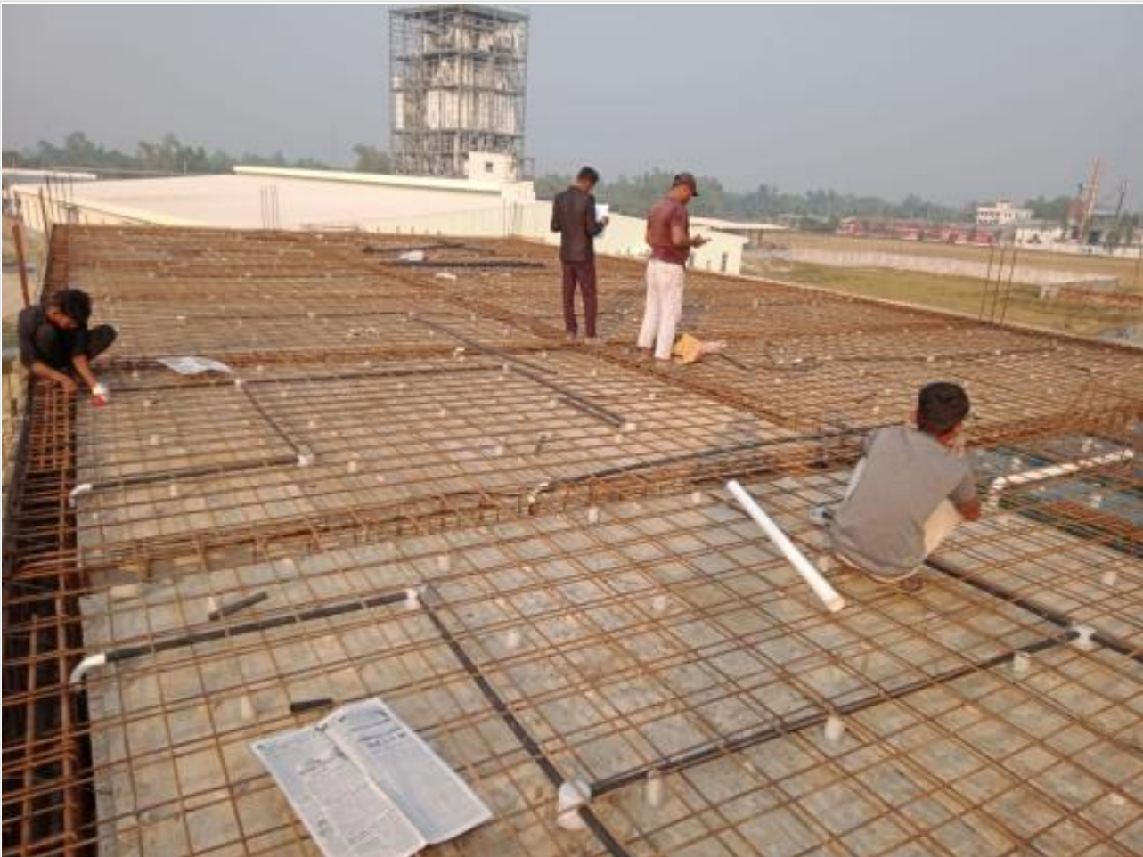
Dormitory-3rd Floor Slab Electrical Pipe on 18-12-23
