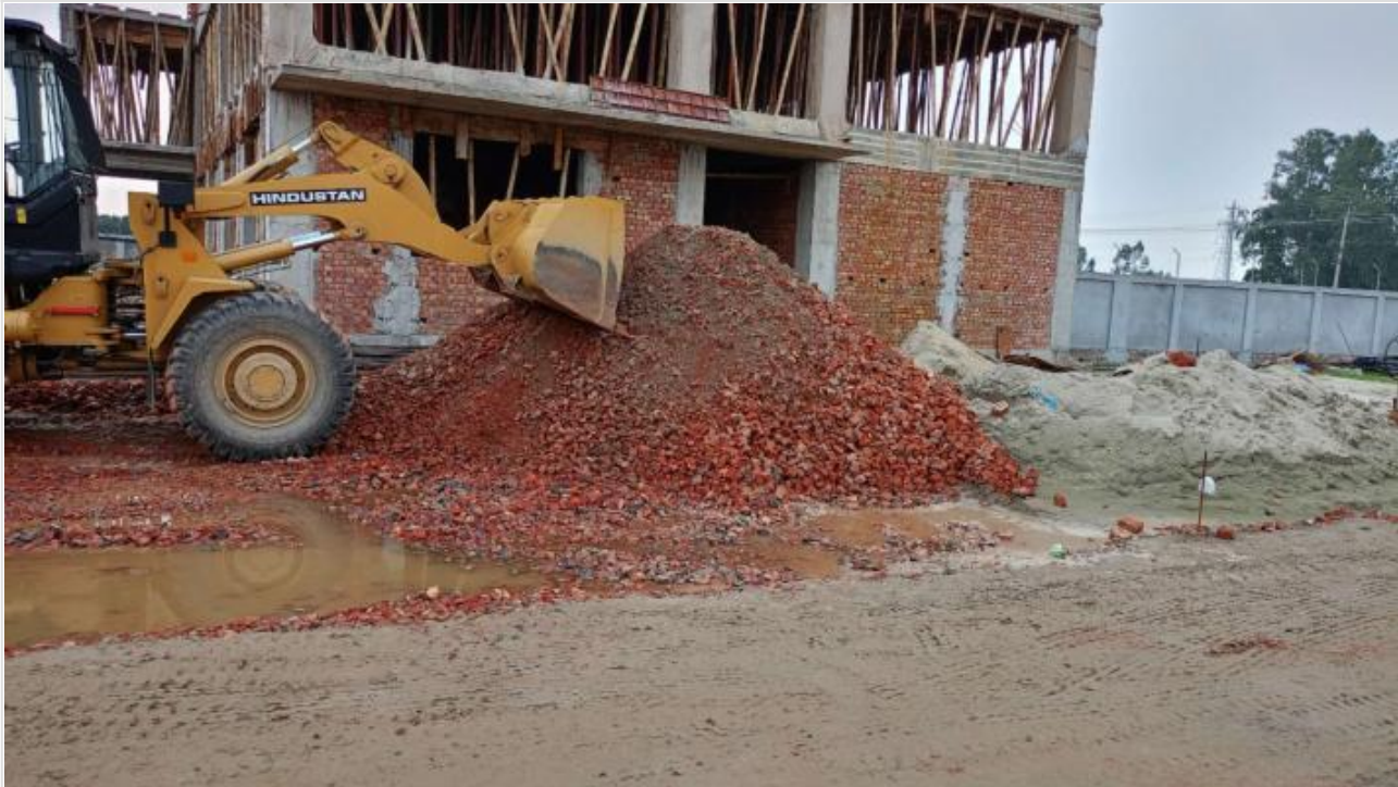
Sub-base-Khoa unloading on 14-08-23
