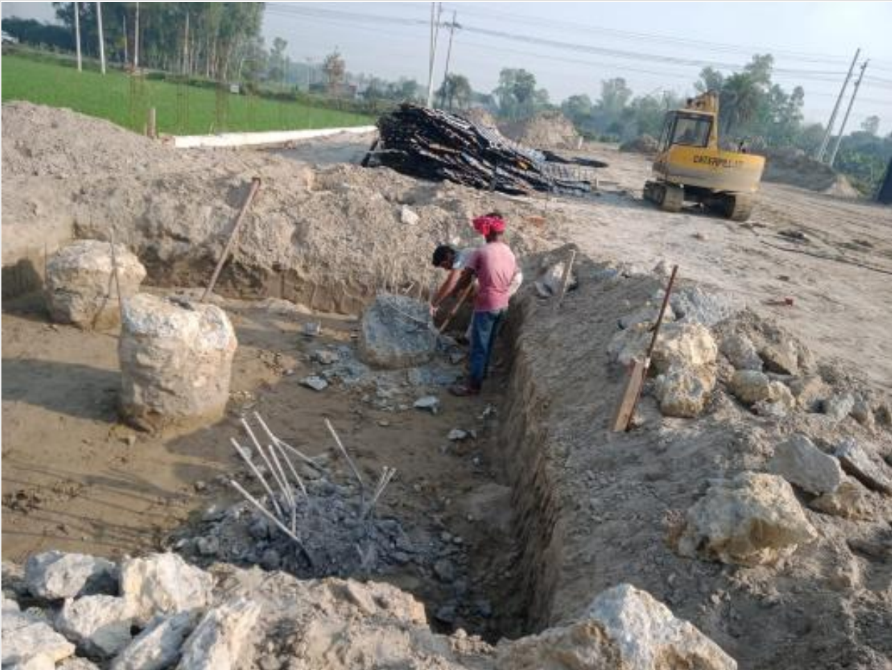
Pile head breaking on 28-03-23
