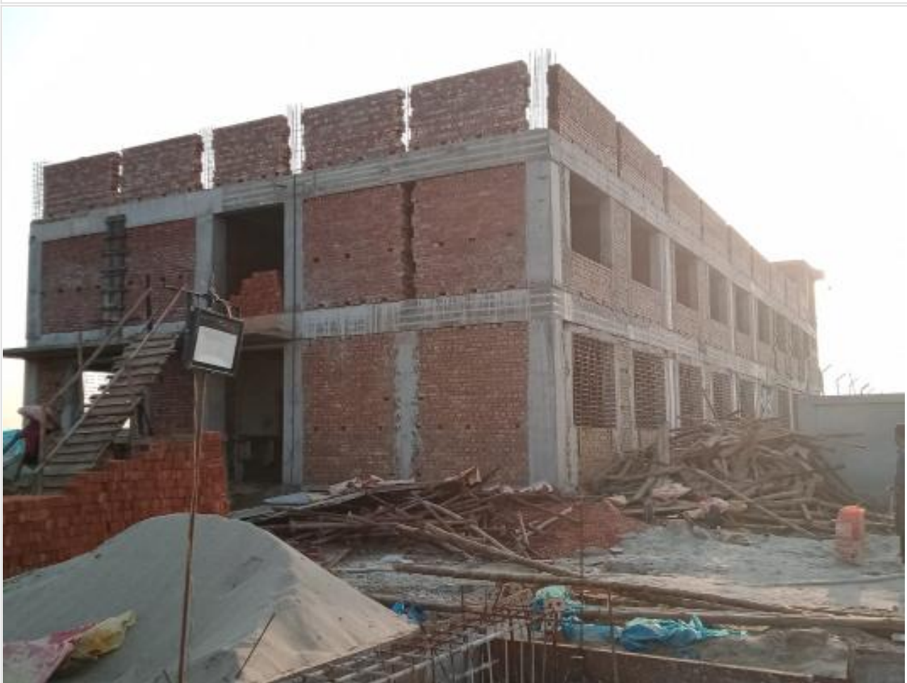
Comp. Bldg work on 15-09-23
