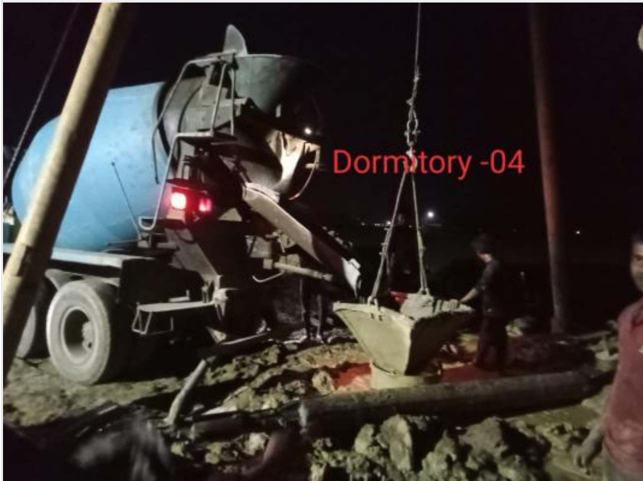
Ready mix concreting of pile on 26-03-23
