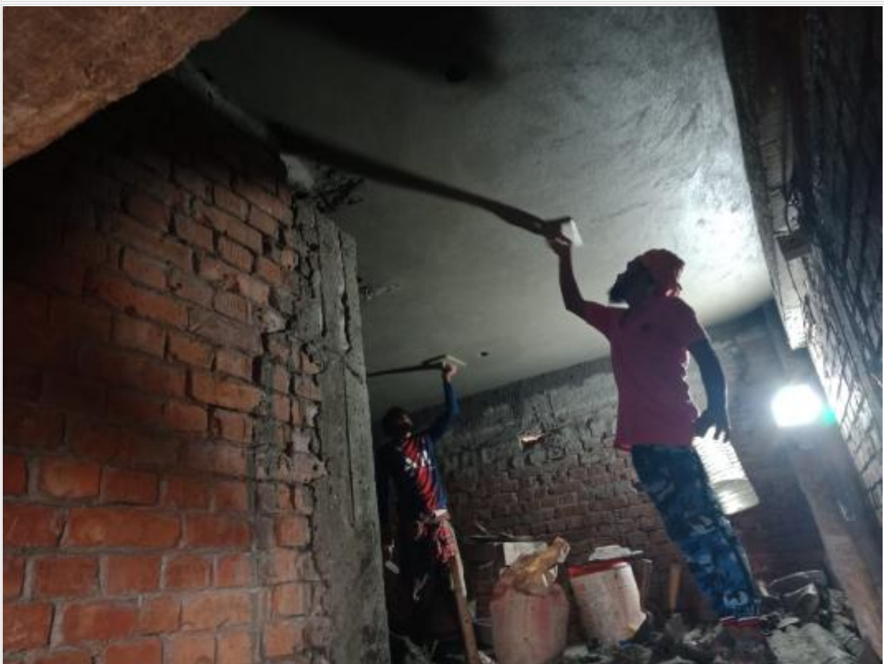
Dorm. Bldg. Ceiling Plaster on 01-11-23
