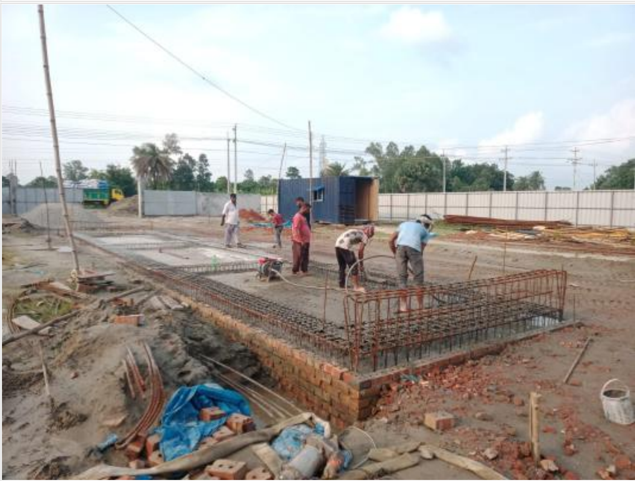
Weighing Bridge Concreting on 23-08-23
