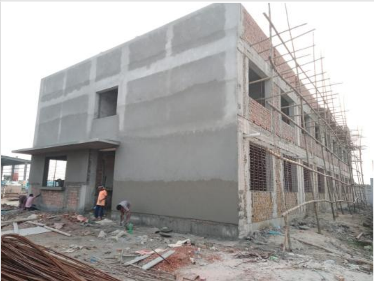
Comp. Bldg. Outside plaster work on 15-10-23
