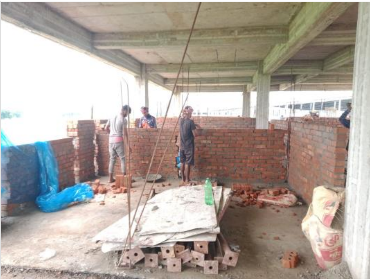
Dorm. Bldg Brick work on 07-10-23
