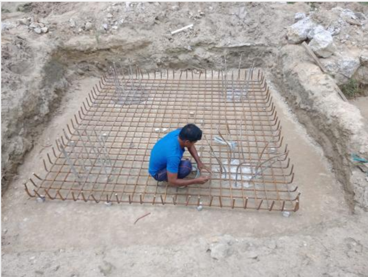
Dorm. Bldg. Pile cap rebar binding on 22-05-23
