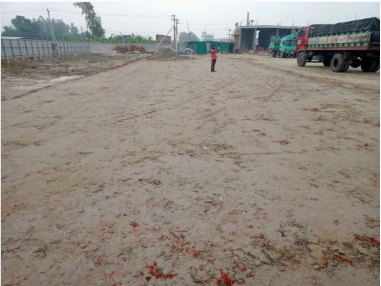
Road work on 13-09-23
