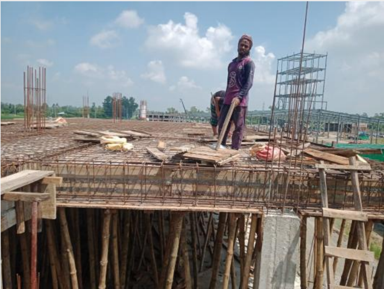
Comp. Bldg. FF Brick work on 10-09-23
