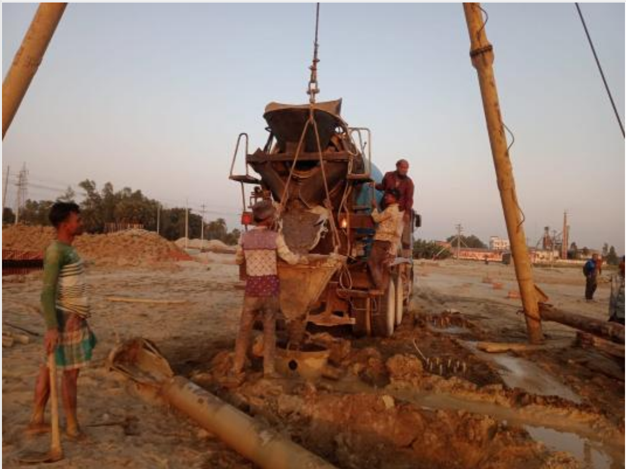
Ready mix concreting of pile on 13-02-23
