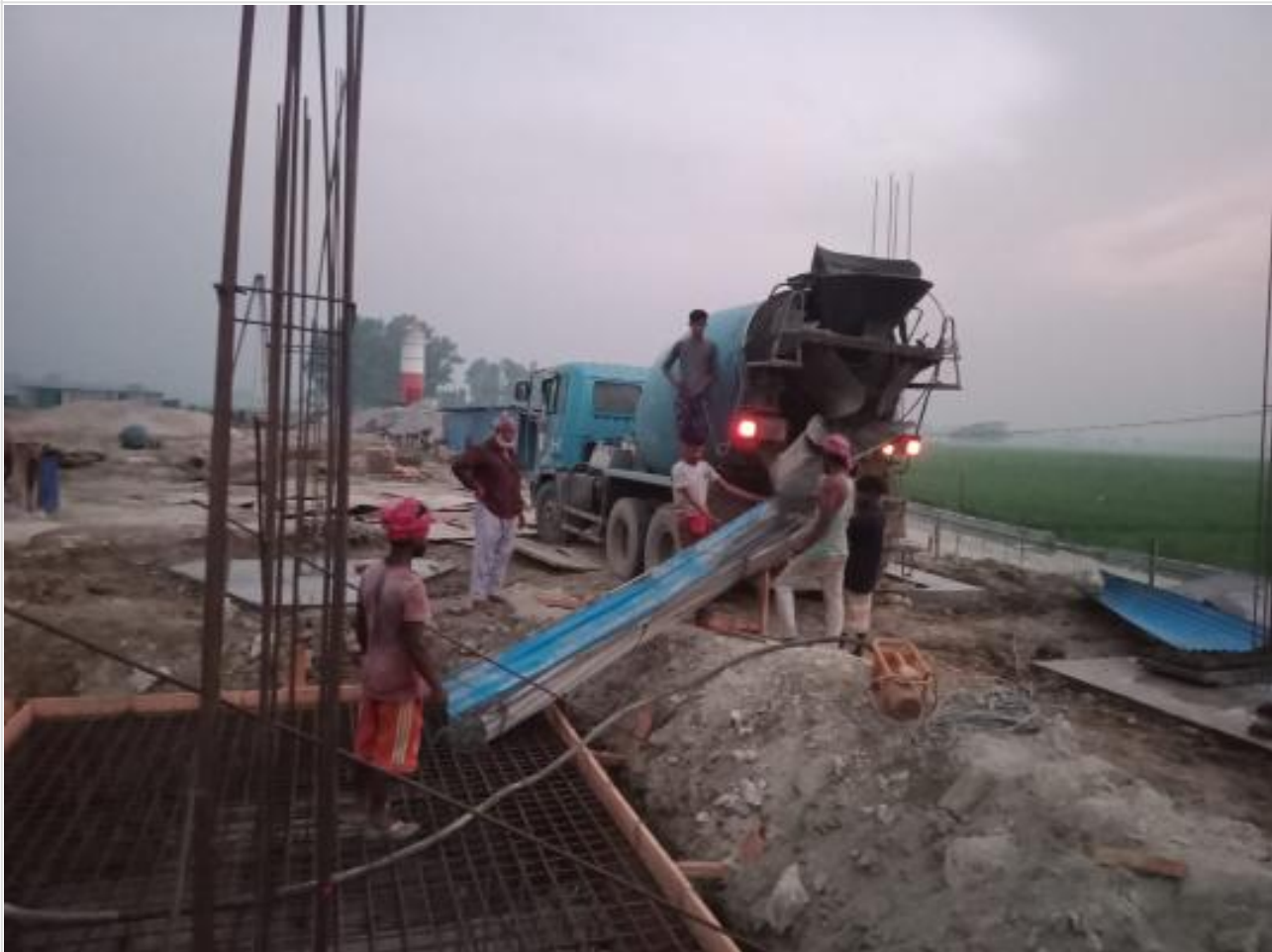
Pile Cap concreting. on 15-04-23
