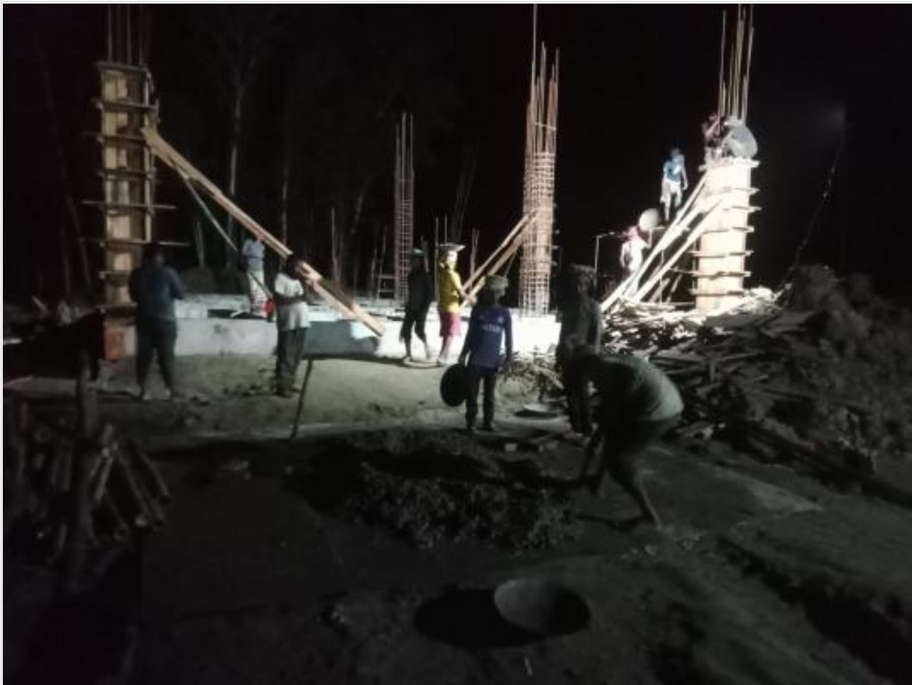
Dorm. Bldg. Column casting on 18-06-23
