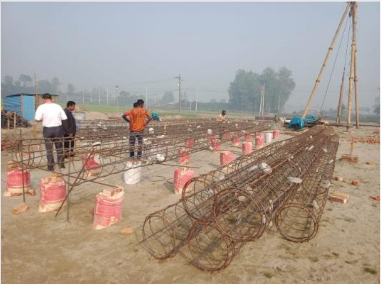
Pile Re-bar Work on 12-02-23
