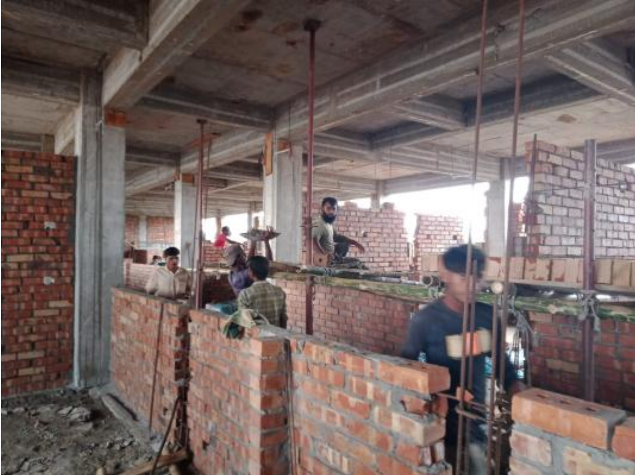
Tie column work at brick wall on 02-08-23
