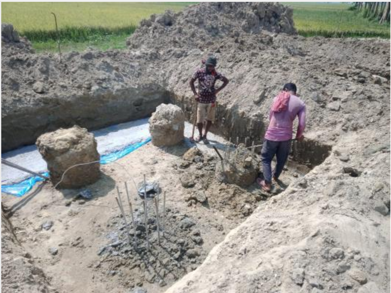
Dorm. Bldg. pile head breaking on 10-05-23
