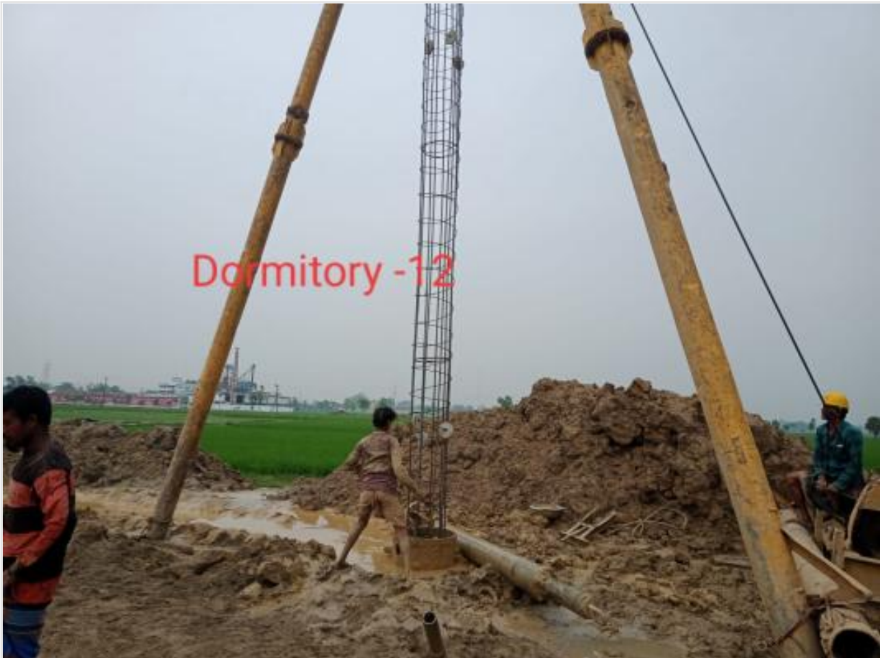
Dorm. Bldg. 10th pile concreting on 30-03-23
