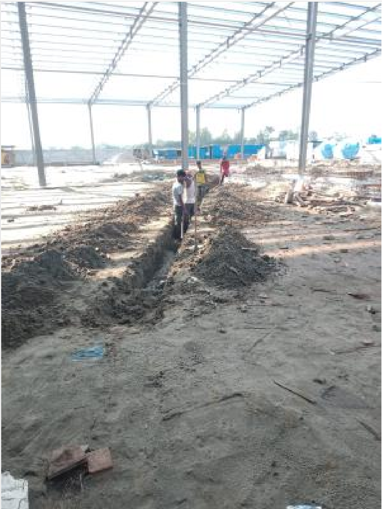
Earth cutting power cable laying on 28-09-23
