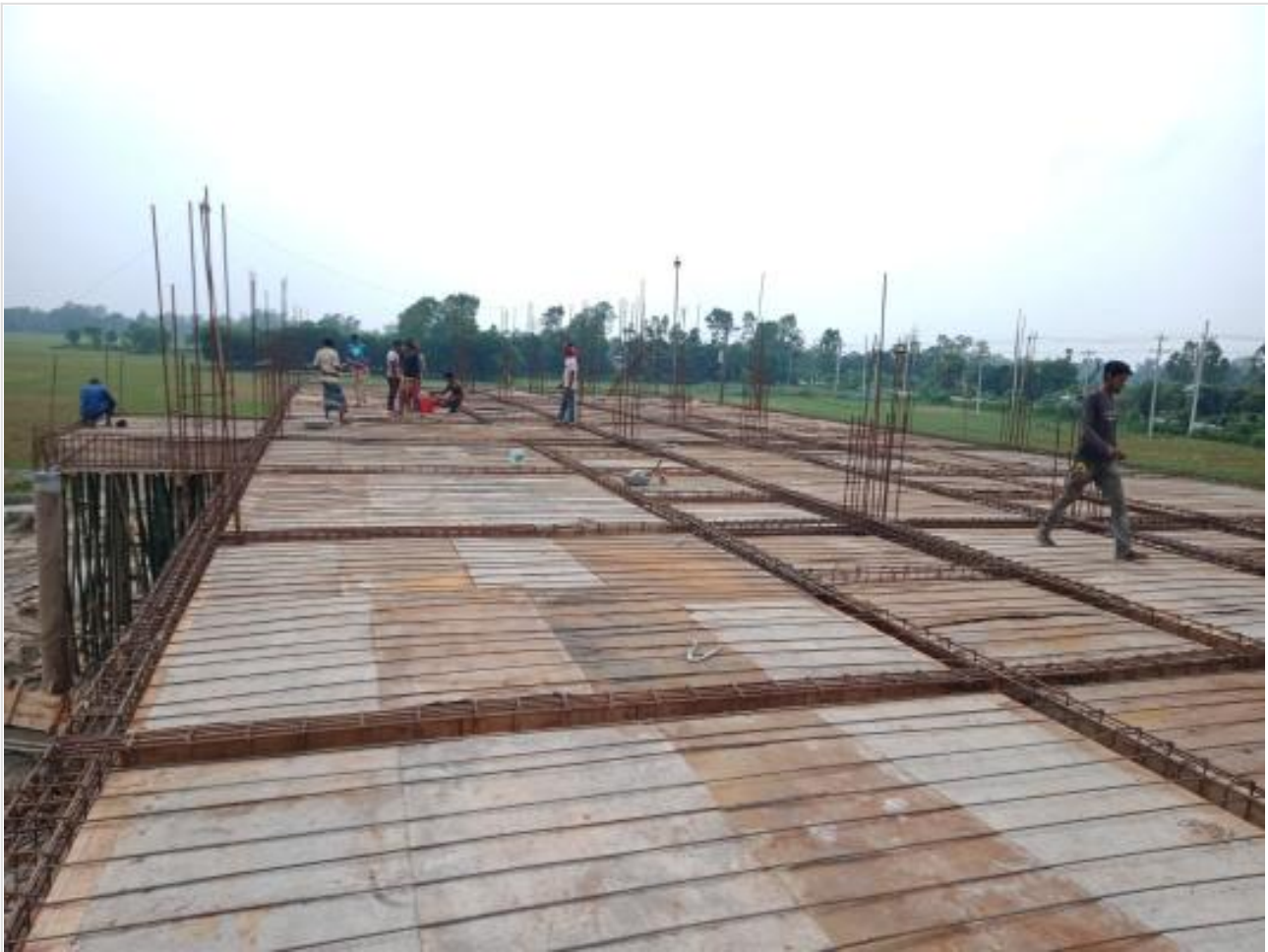
Comp. Bldg. Slab beam shuttering on 15-06-23
