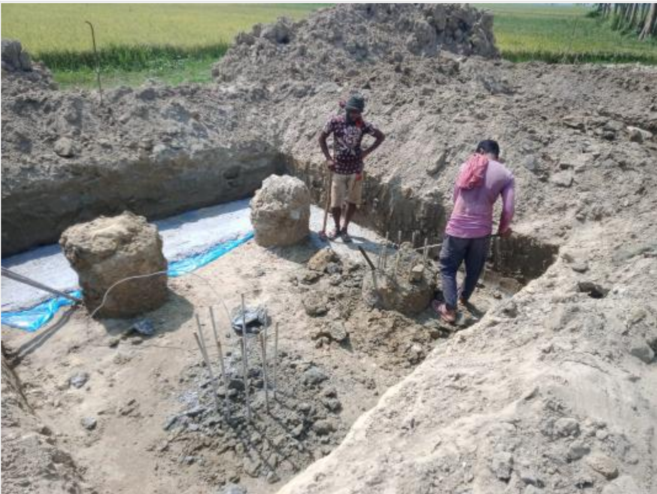
Dorm. Bldg. pile head breaking on 10-05-23
