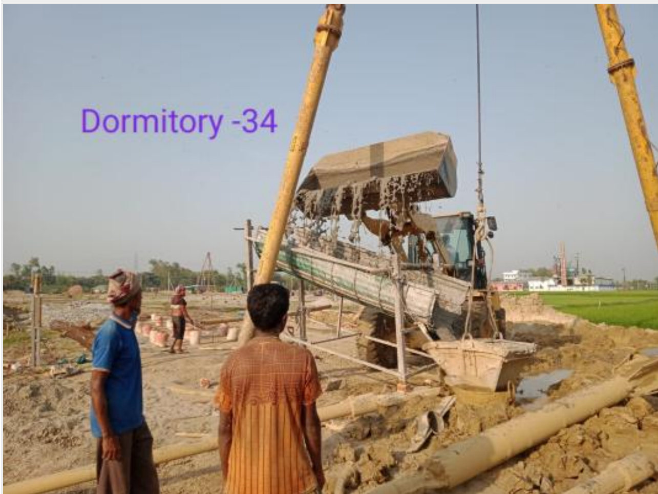
Dorm. Bldg. 32nd pile concreting on 09-04-23
