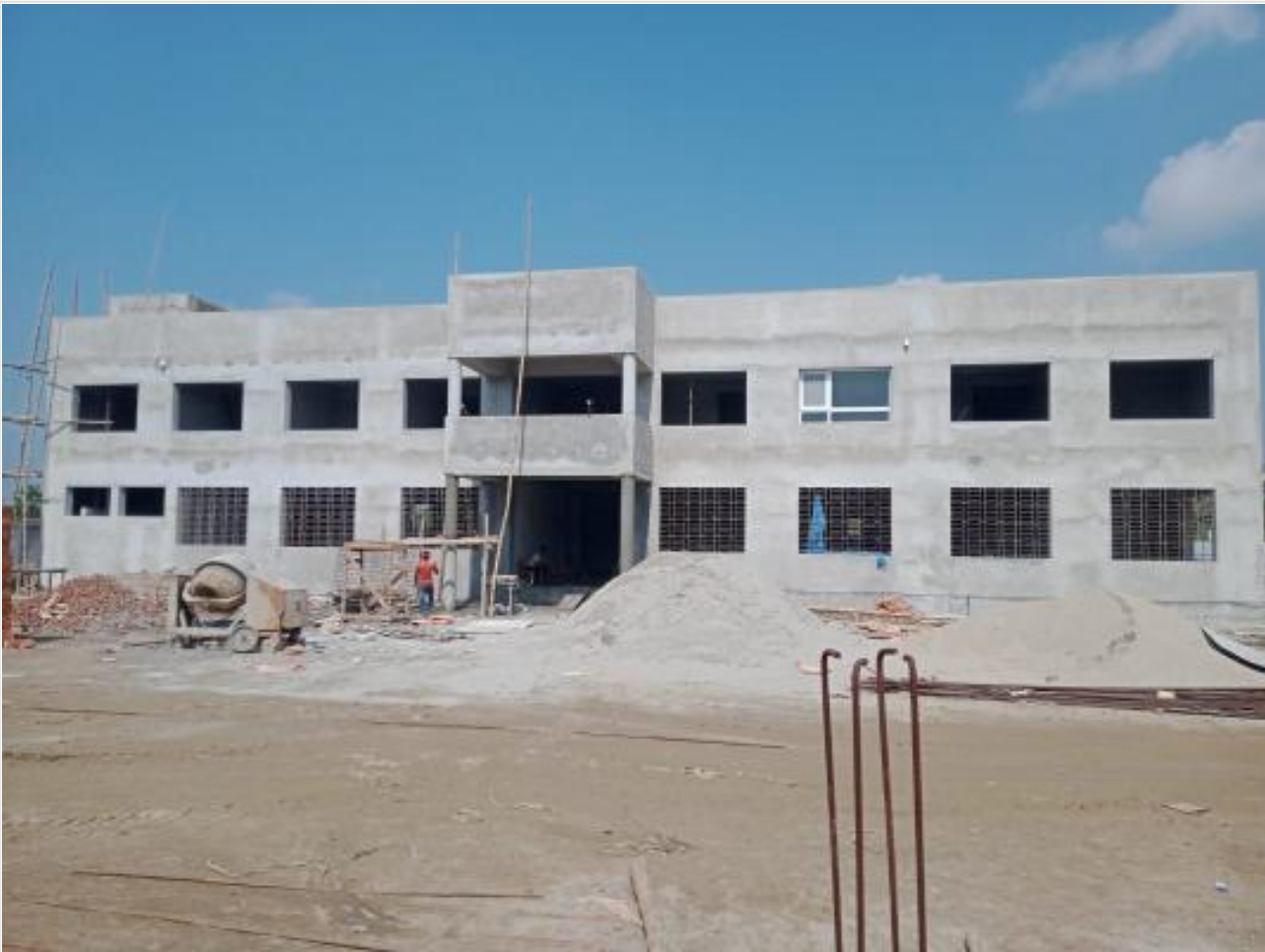
Comp. Bldg. on 26-10-23
