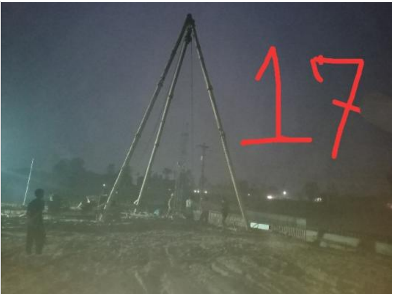
Com. Bldg. 17th Pile Boring on 21-02-23
