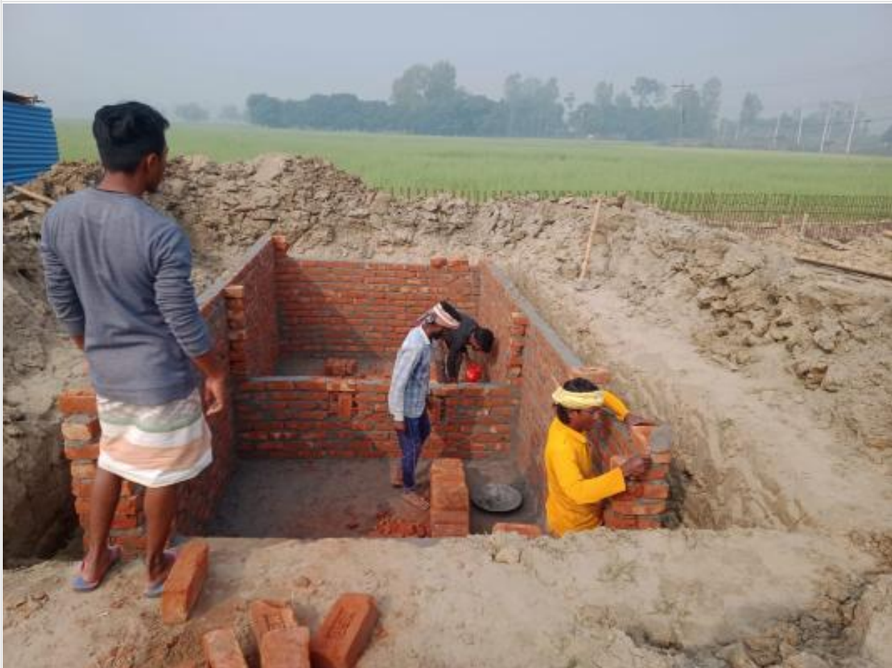
Mud Tank making on 06-02-23
