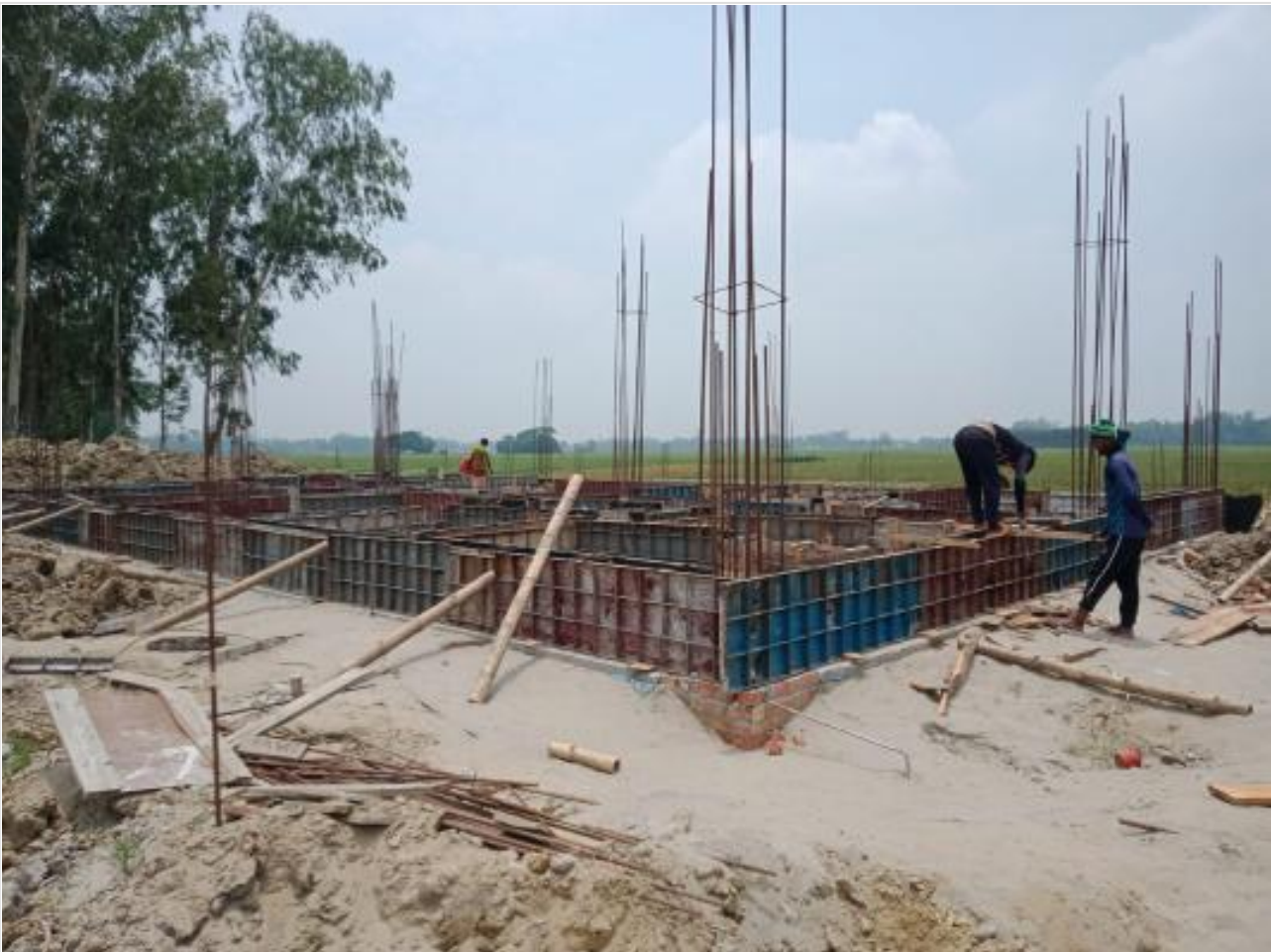
Dorm. Bldg. GB shuttering on 09-06-23
