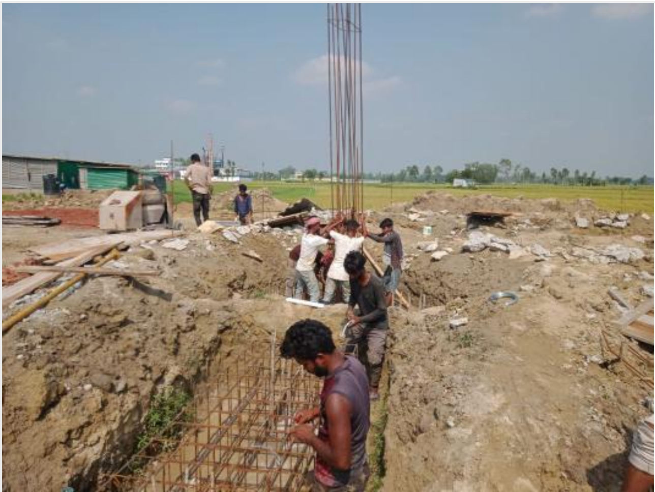
Dorm. Bldg. Pile cap rebar binding on 24-05-23
