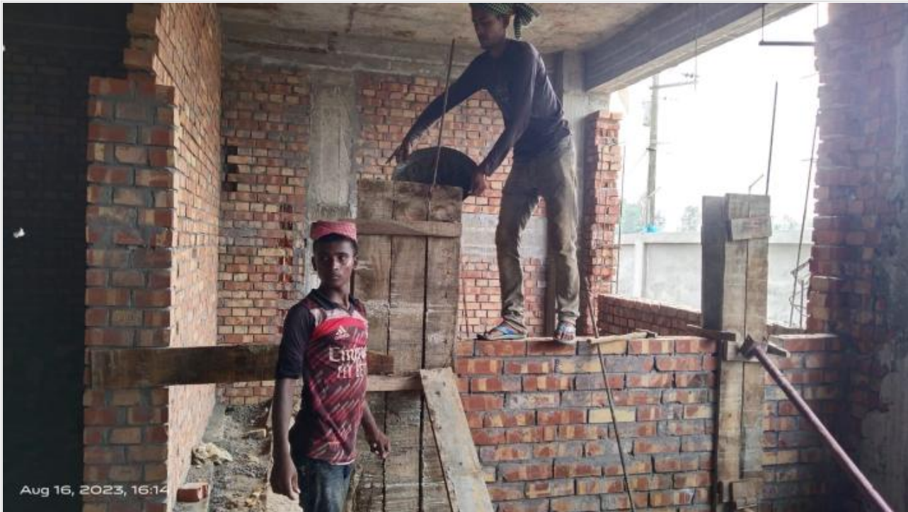
Comp-GF Column Concreting on 16-08-23
