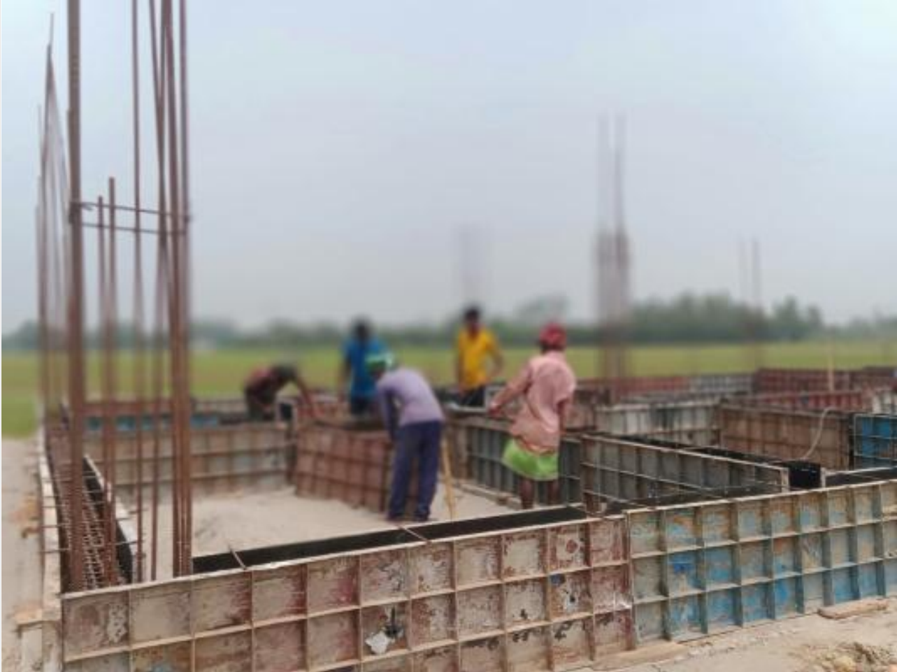
Dorm. Bldg. GB shuttering on 09-06-23
