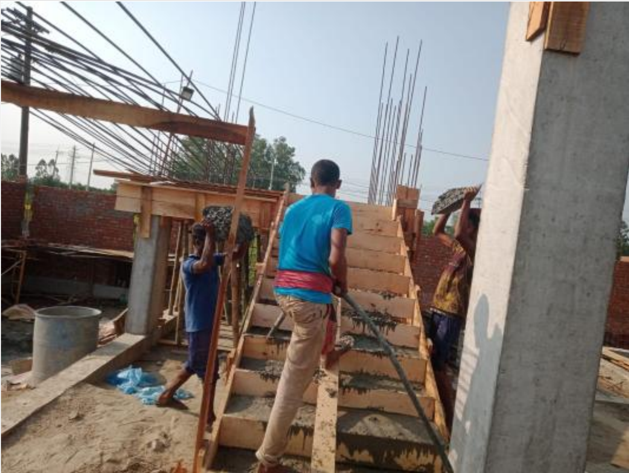
1st flight stair casting on 05-06-23
