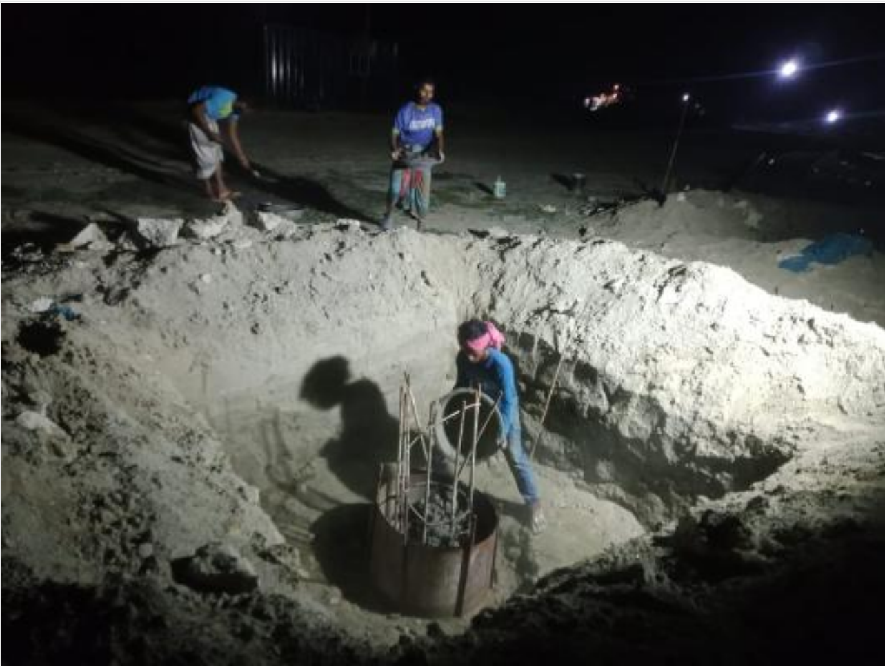
Gate pile Cap cc work on 08-05-23
