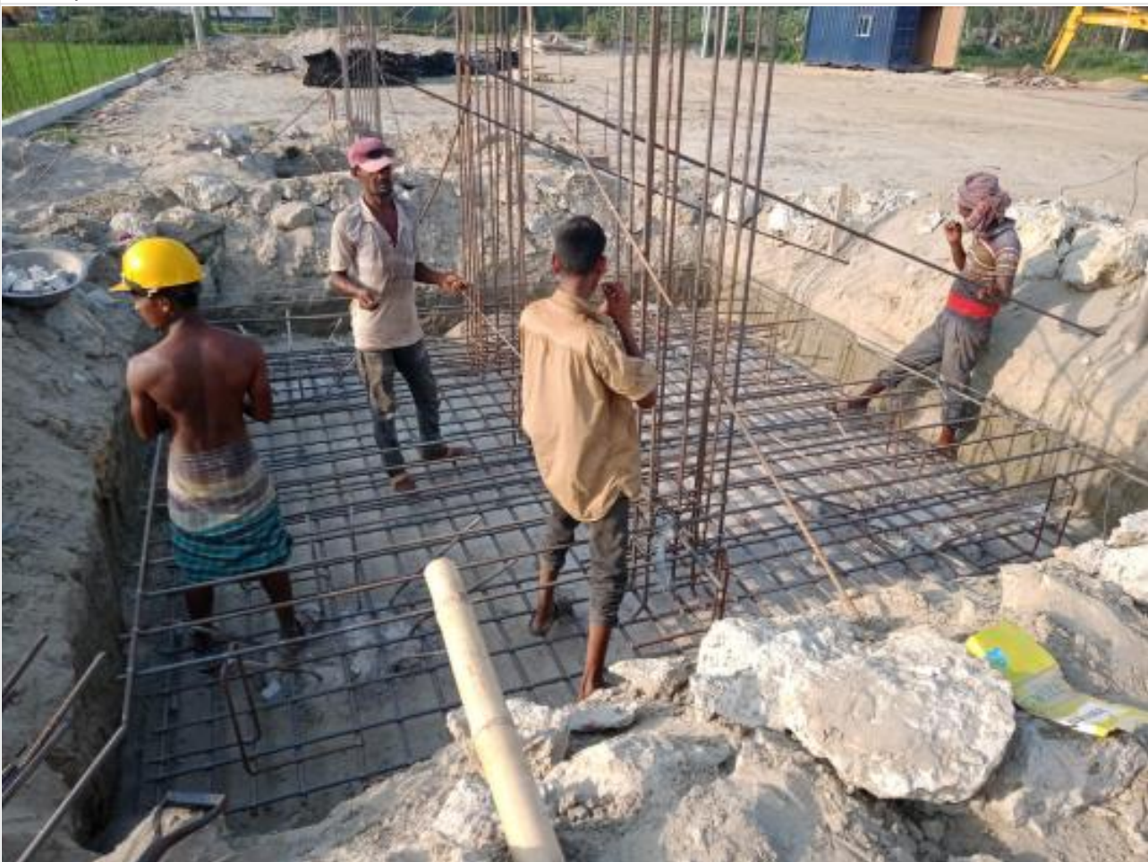
Pile cap rebar work on 14-04-23
