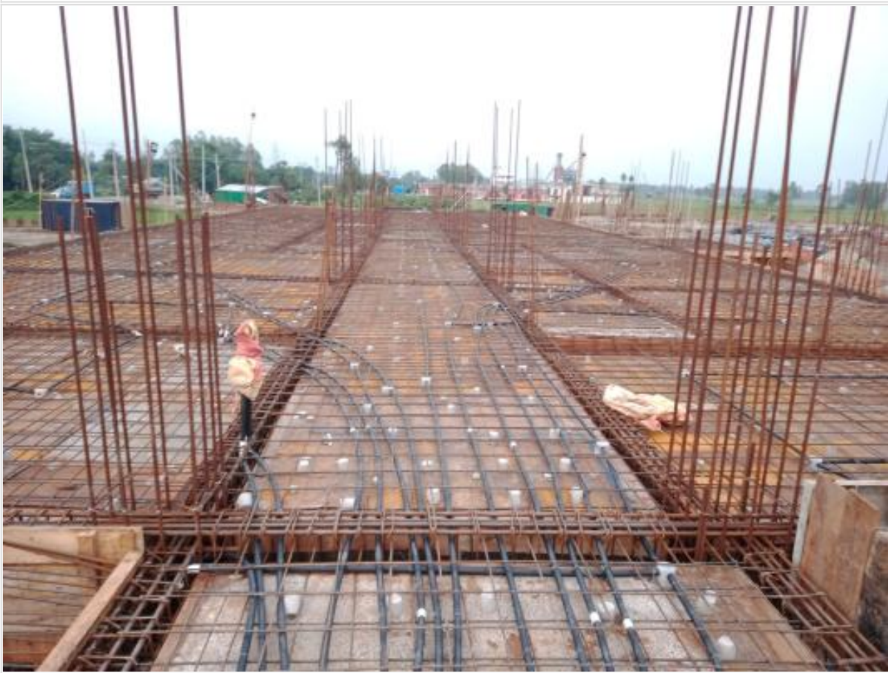
Comp. Bldg. Slab Ready for Concrete on 22-06-23
