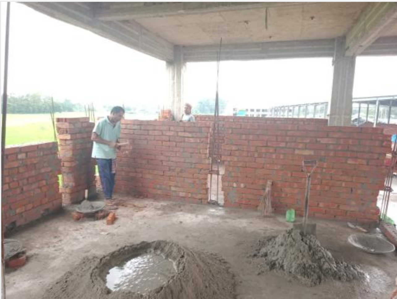
Dorm. 1st floor brick work on 04-10-23
