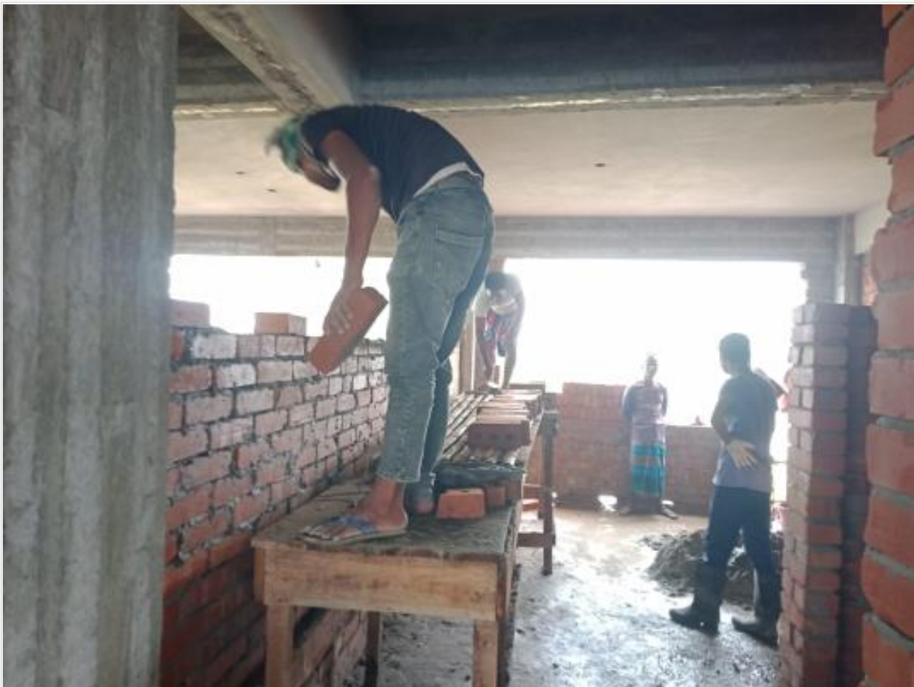
Comp. Bldg. 1st floor brick wall on 04-09-23
