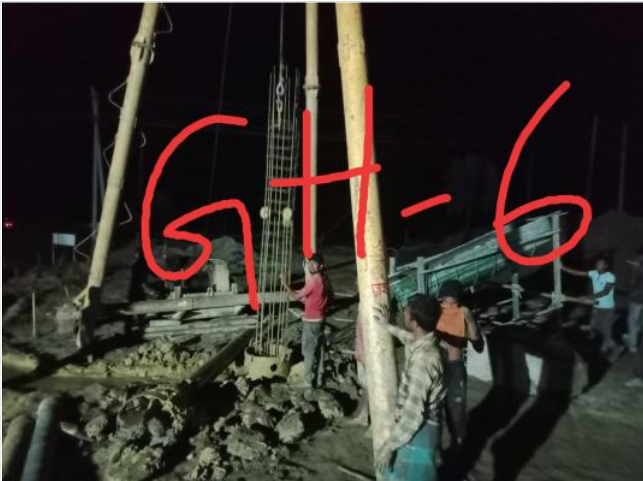
Guard House pile concreting by RMC on 19-03-23
