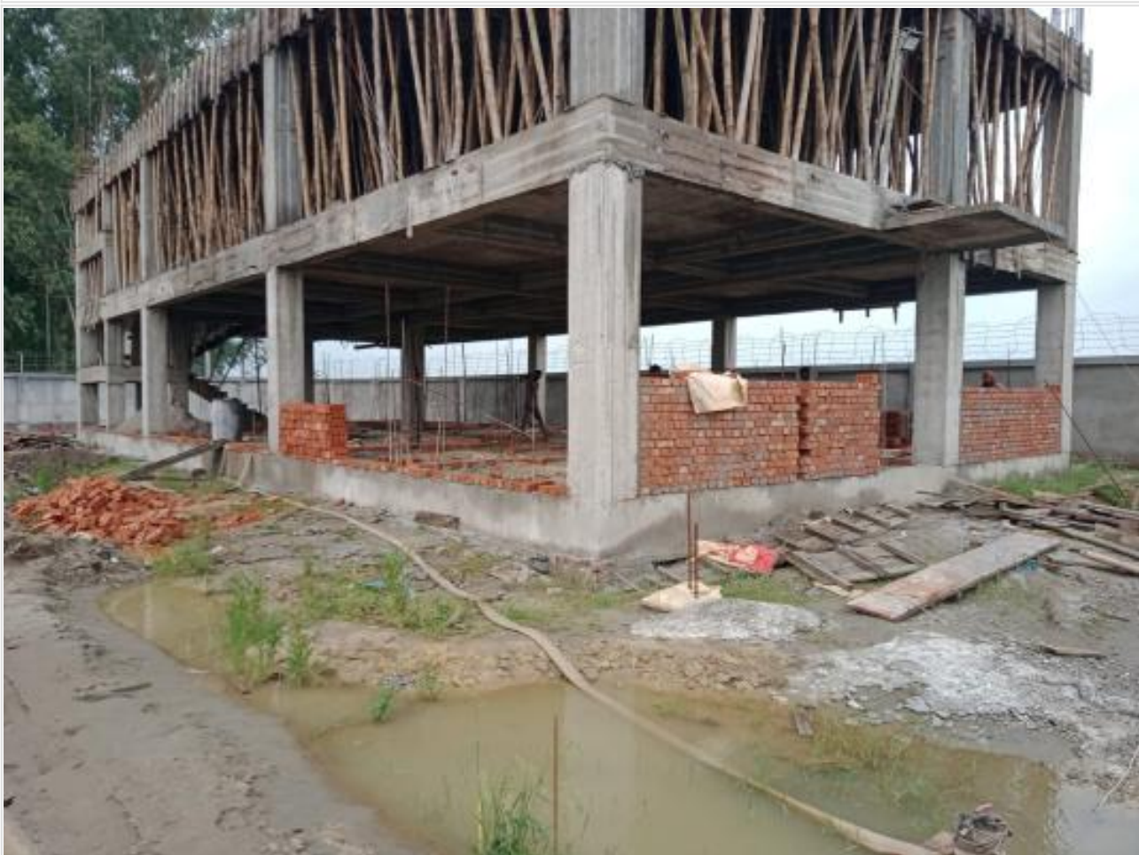
Dorm. Bldg GF Brick work on 21-09-23
