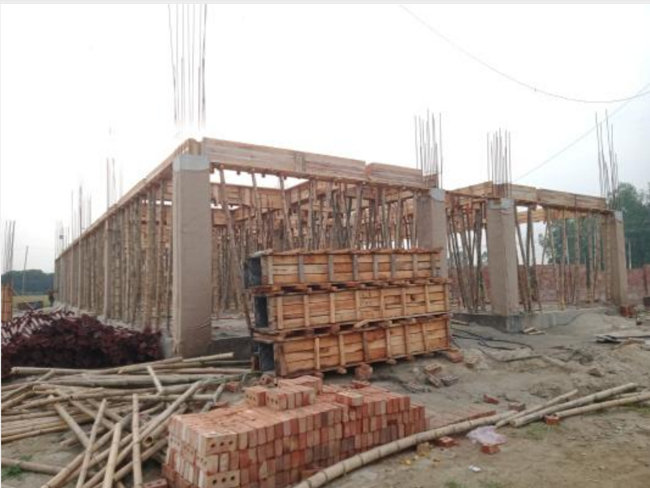
Comp. Bldg. Slab beam shuttering on 07-06-23
