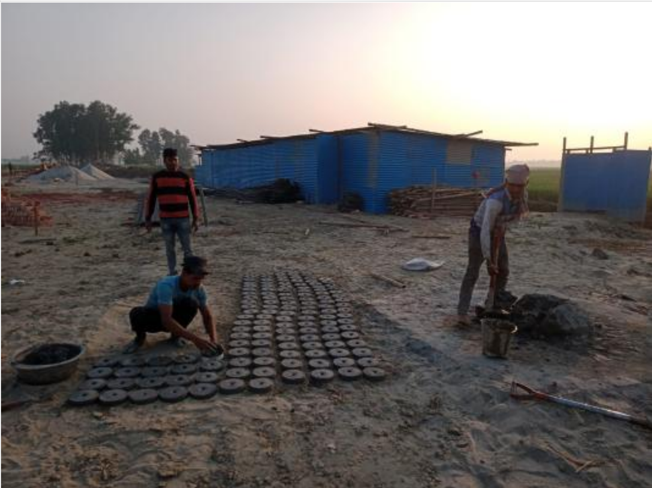
Pile re-bar spacer block making on 02-02-23
