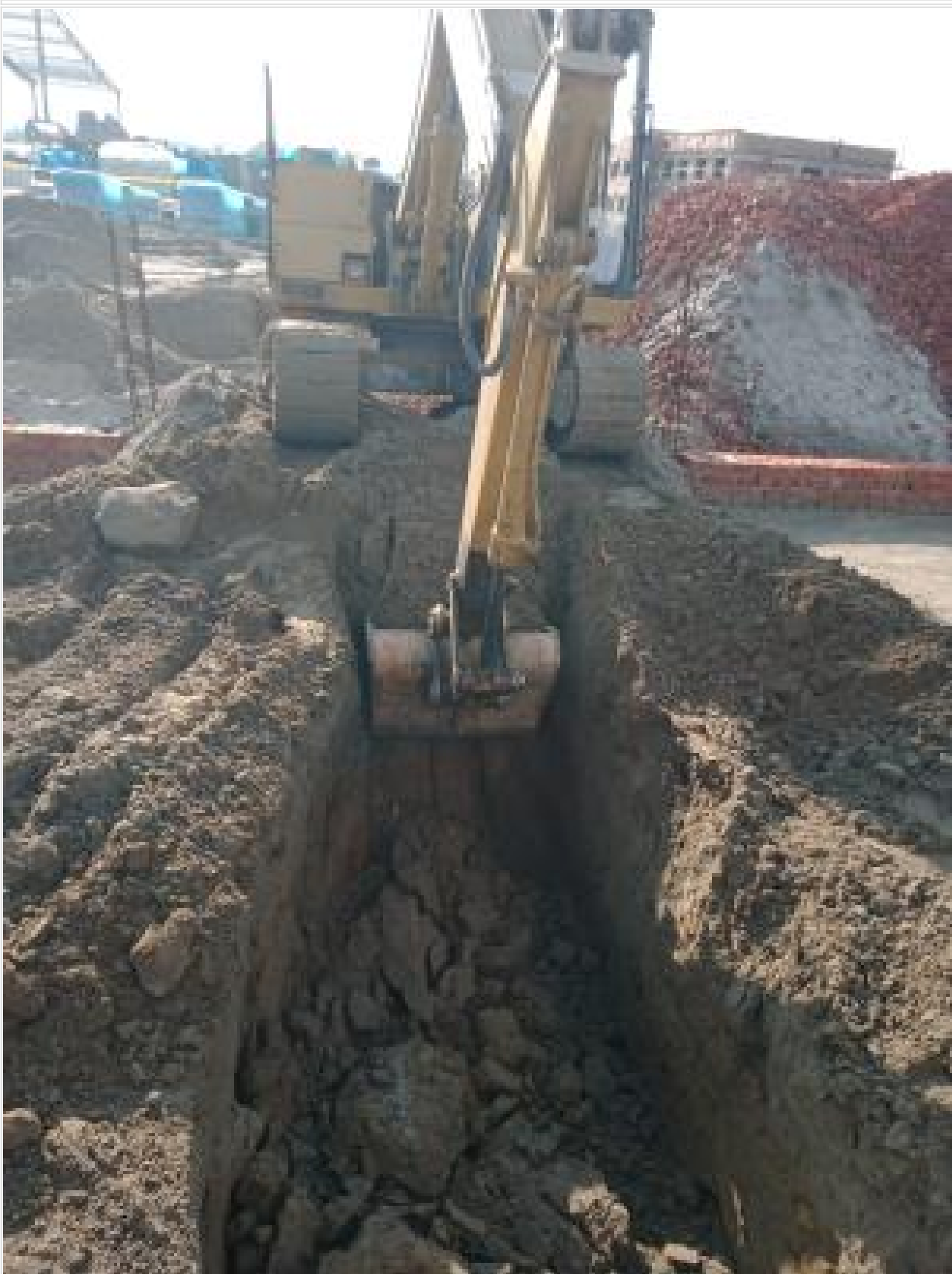
Earth cutting Electric line on 01-10-23
