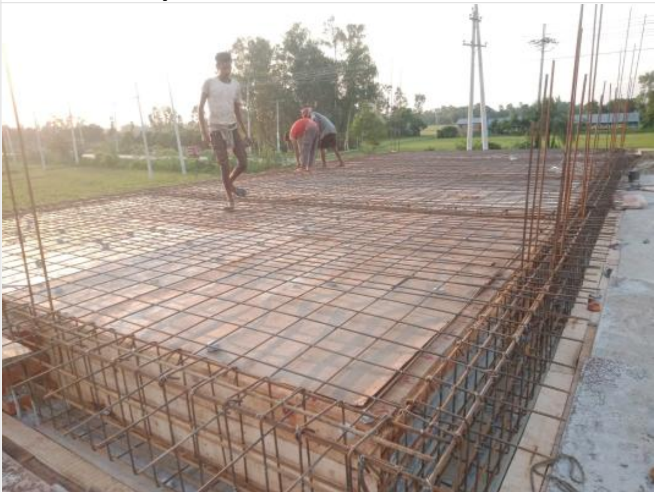
Gate House work on 25-06-23
