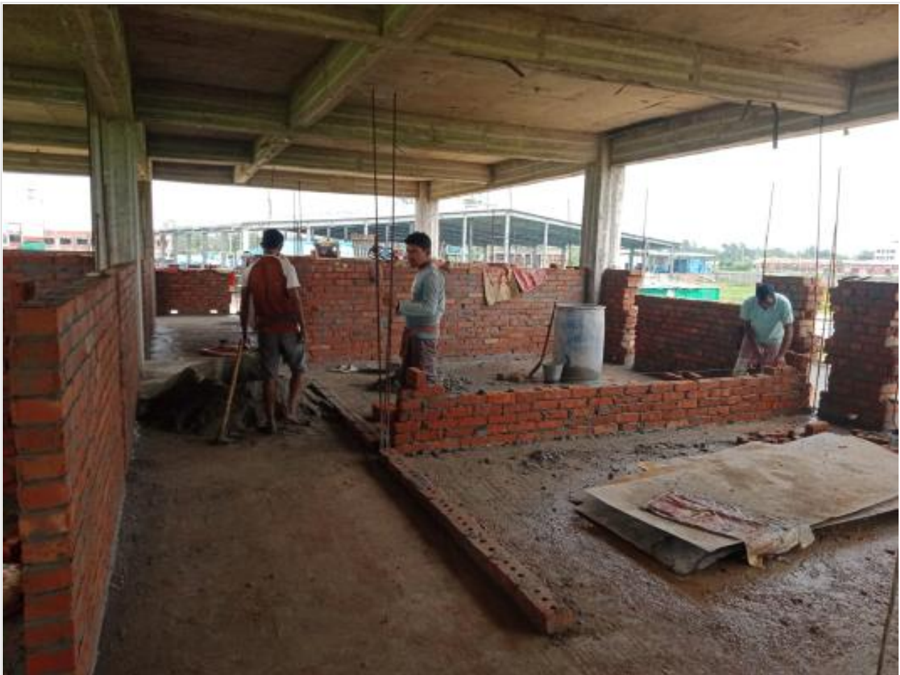
Dorm. Bldg. 1st floor brick work on 06-10-23
