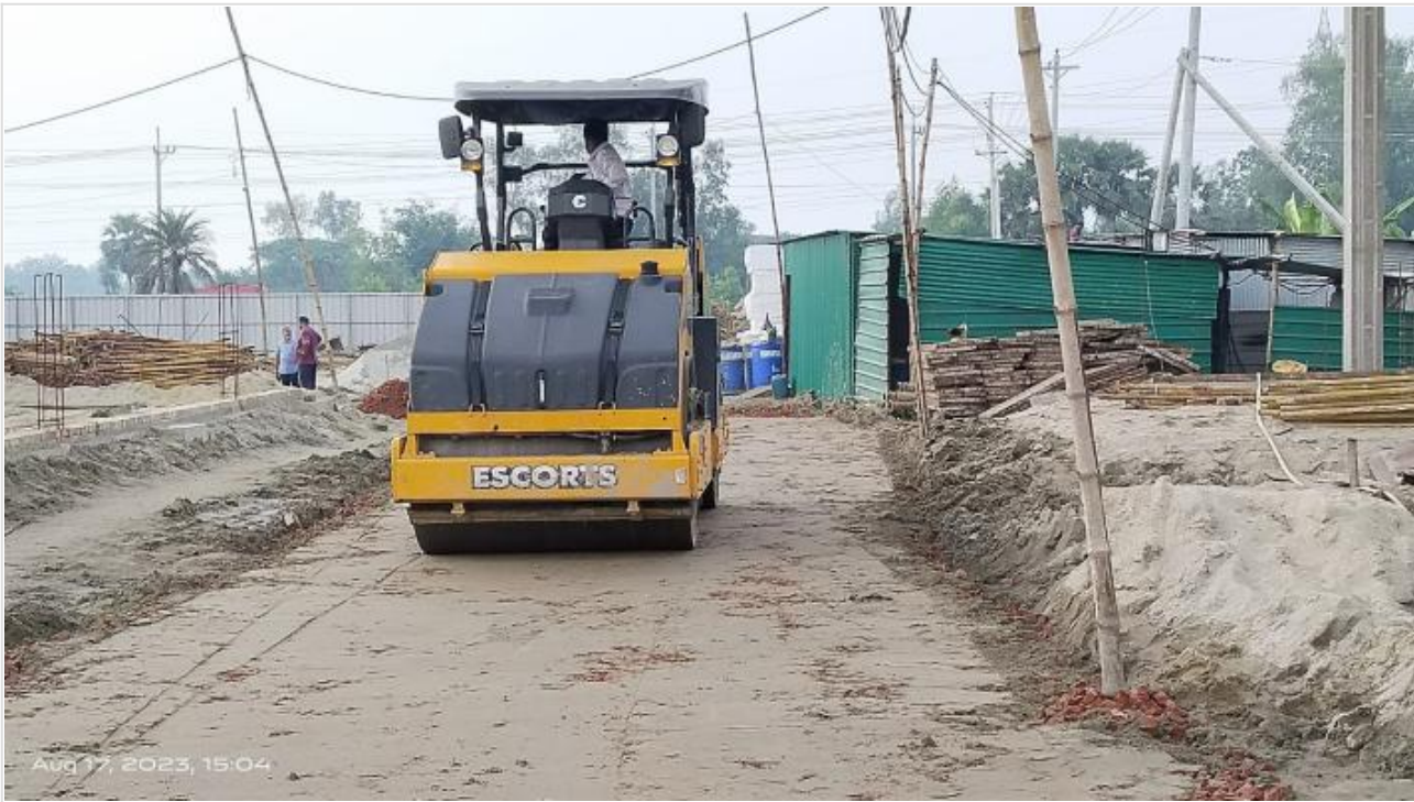
Sub-base Compaction on 17-08-23
