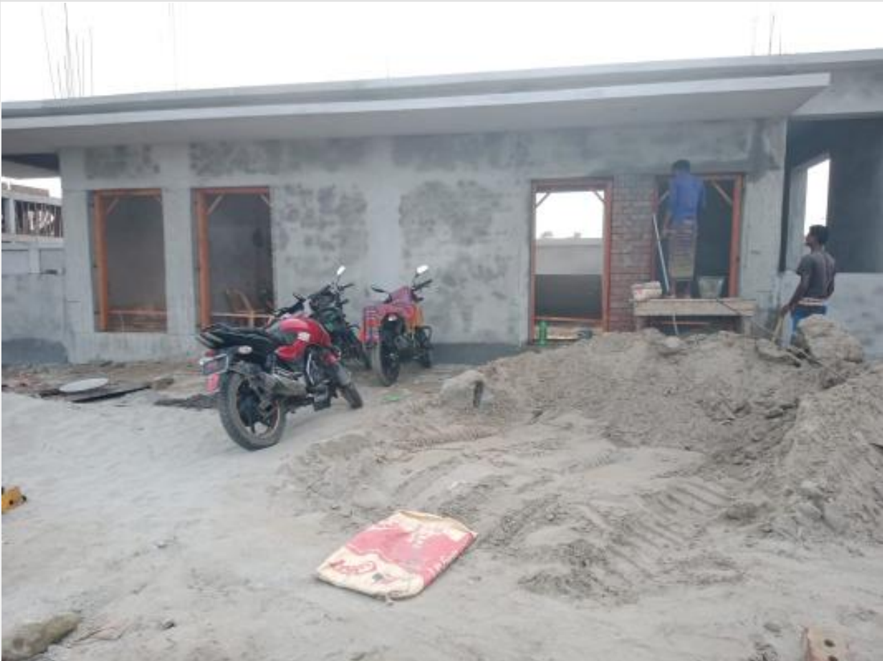
Gate House-Door Frame Fixing on 20-08-23
