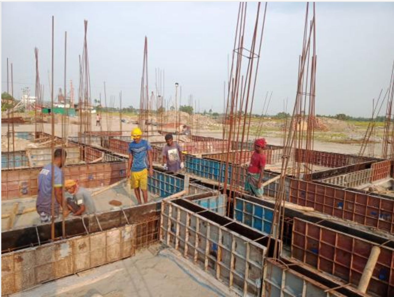
GB Shuttering work on 14-05-23
