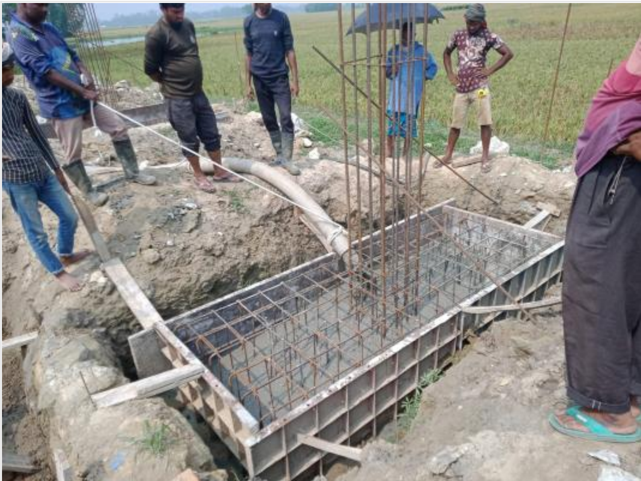
Dorm. Bldg pile cap casting on 28-05-23
