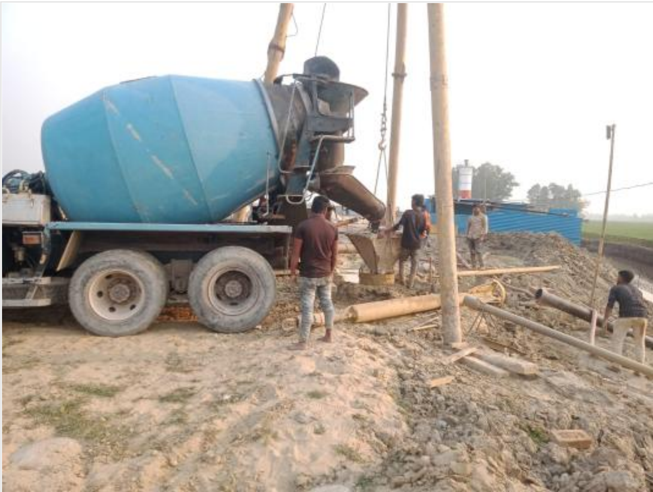
Ready mix concreting of pile on 16-02-23
