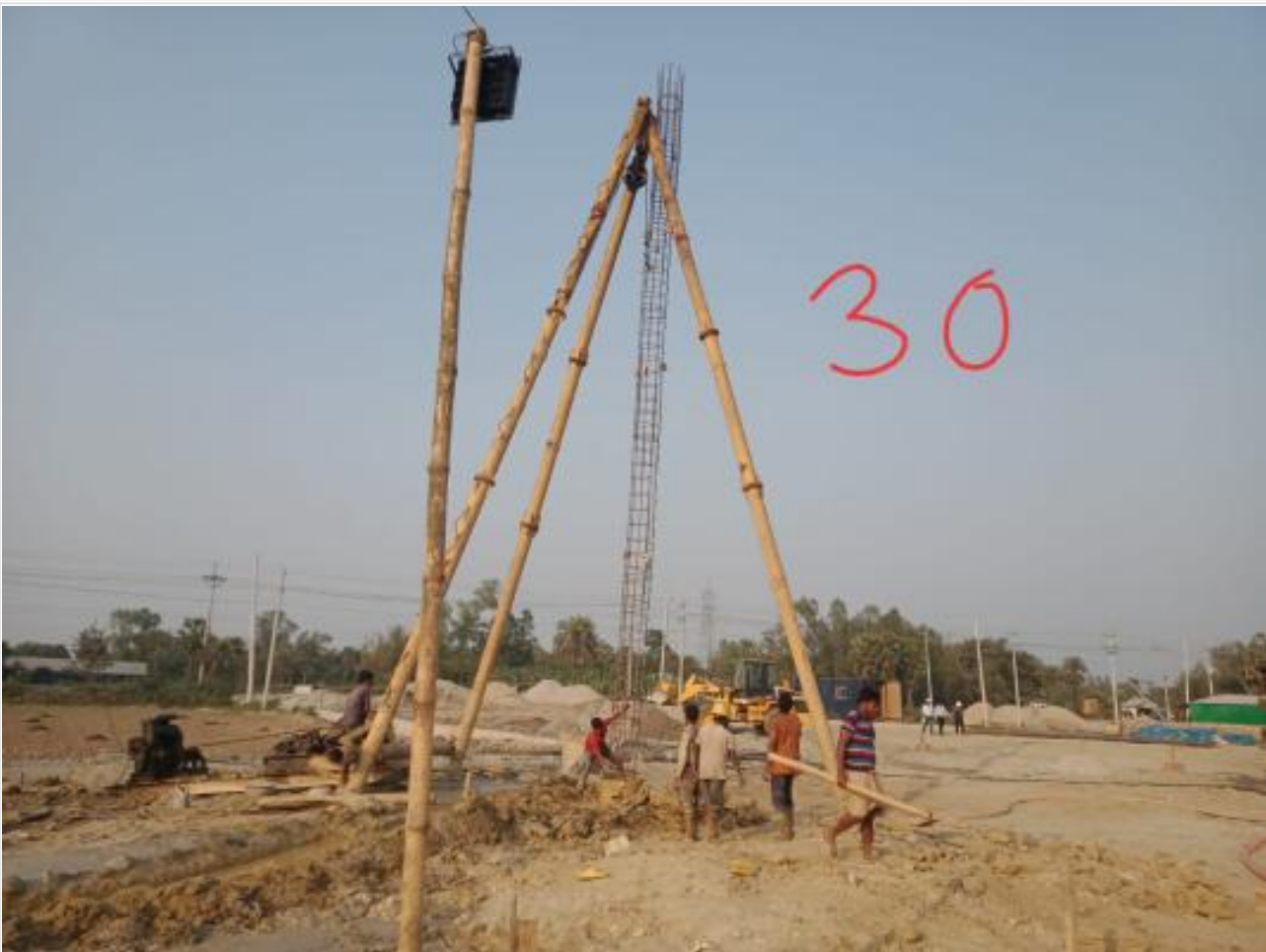
Com. Bldg. 30th pile boring on 26-02-23
