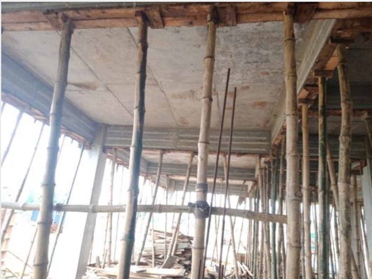
Comp. Bldg. Slab shutter opening on 12-07-23
