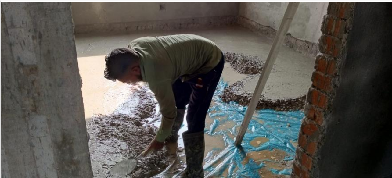
Dorm. Bldg. GF Concreting on 10-11-23
