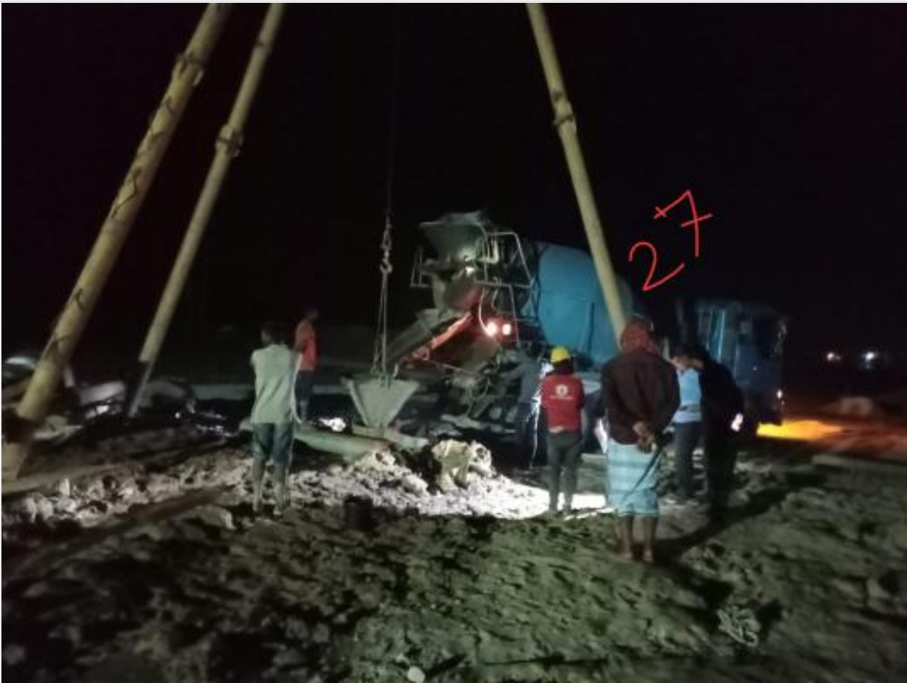
Ready mix concreting of pile on 25-02-23
