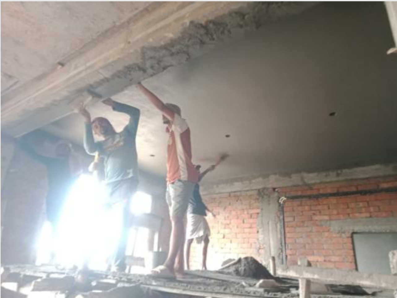
Ceiling plaster on 25-10-23
