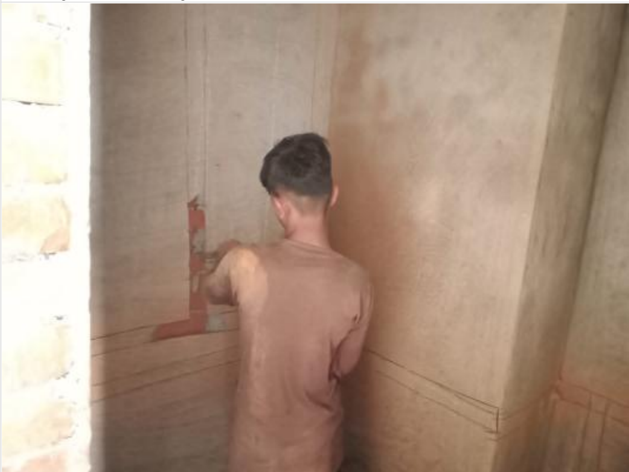
Sanitary group cutting on 06-11-23
