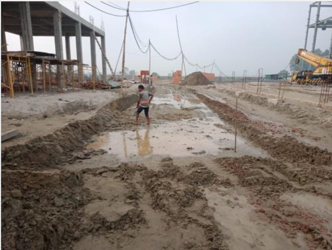
Road-Excavation-box cutting on 16-08-23
