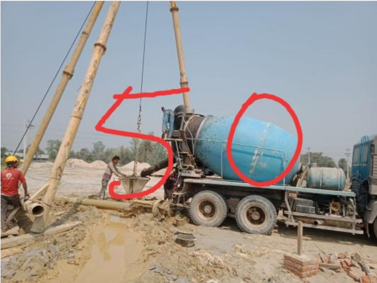
Ready mix concreting of pile on 09-03-23
