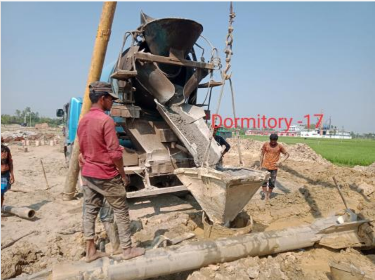
Ready mix concreting of pile on 02-04-23
