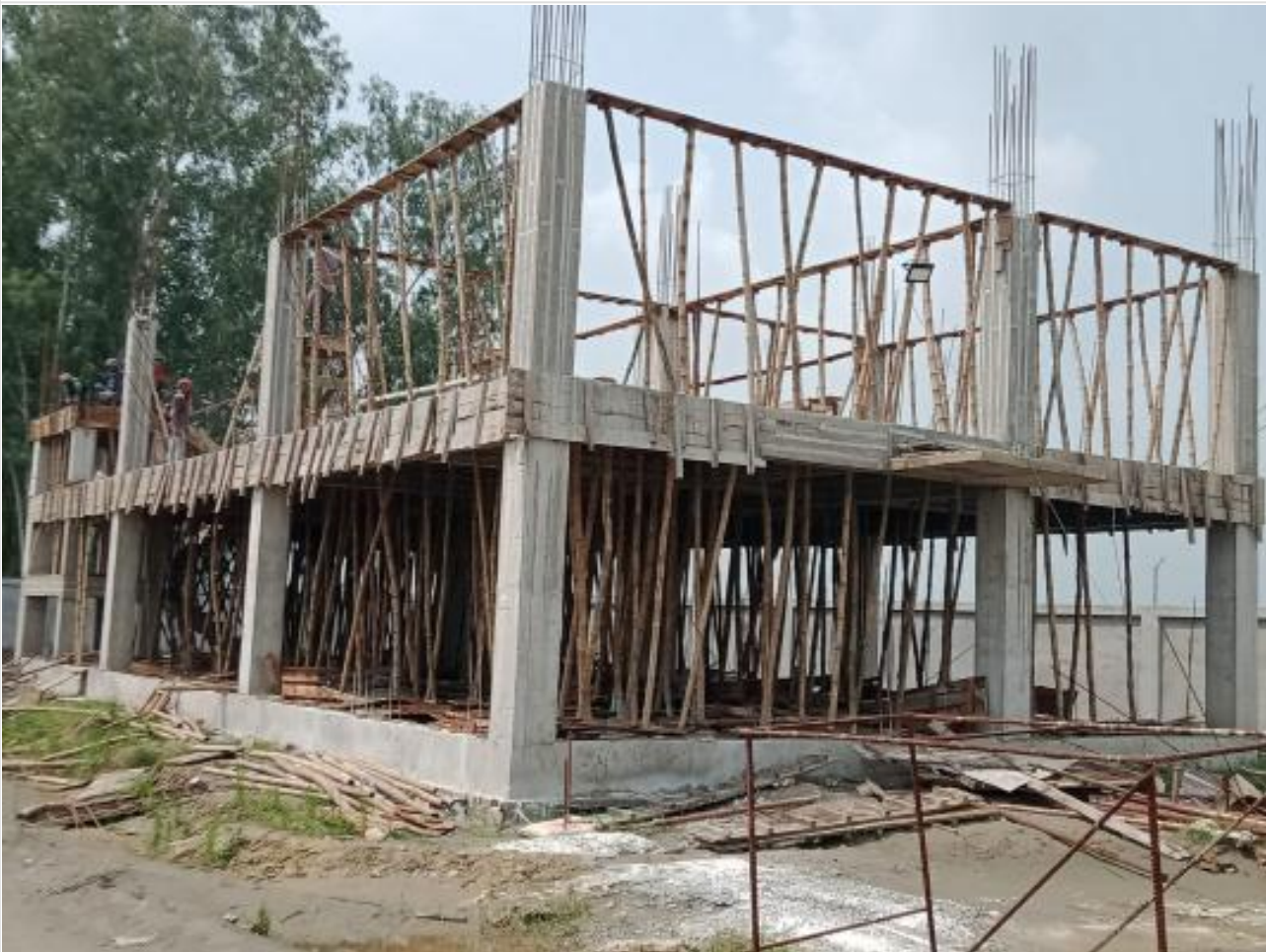
Dorm. Bldg. 2nd floor shuttering on 29-08-23
