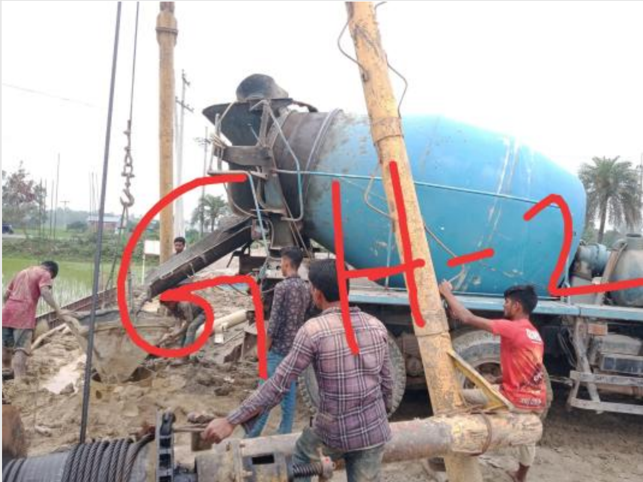
Guard House pile concreting by RMC on 19-03-23
