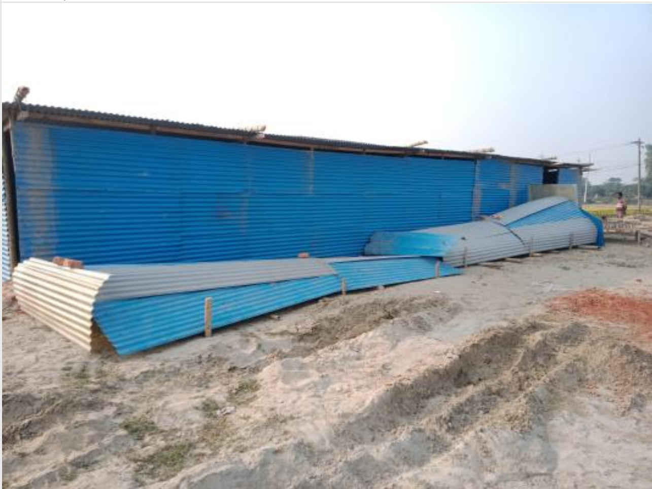
Shed completed on 22-01-23
