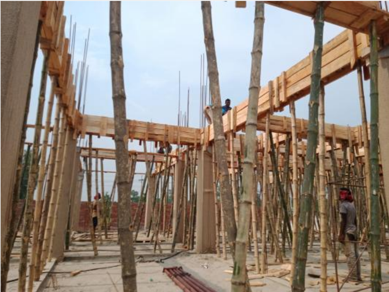
Comp. Bldg. Slab beam shuttering on 07-06-23
