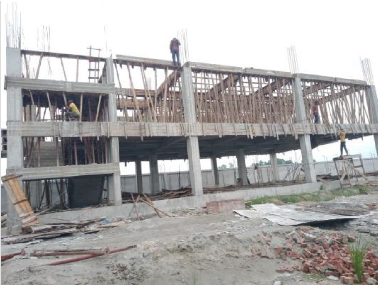
Dorm. Bldg. 2nd floor Shuttering work on 04-09-23
