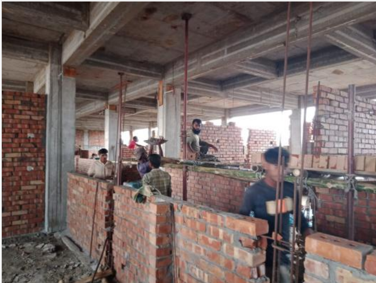
Tie column work at brick wall on 02-08-23
