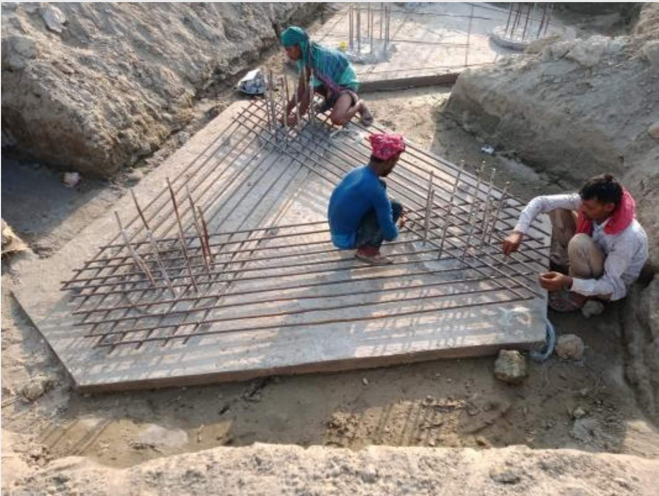
Pile cap work on 14-04-23
