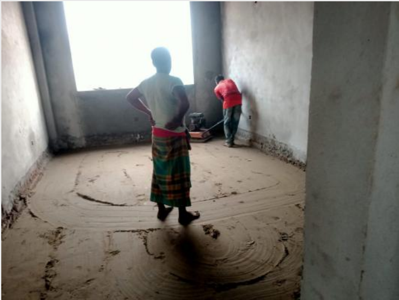
Comp. Bldg floor GF compaction on 11-09-23
