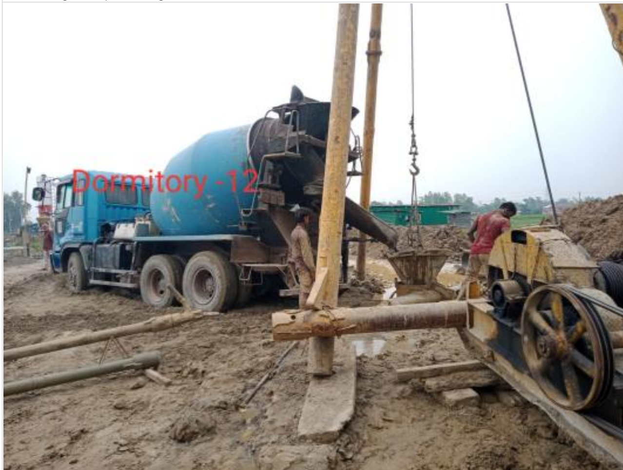
Ready mix concreting of pile on 31-03-23
