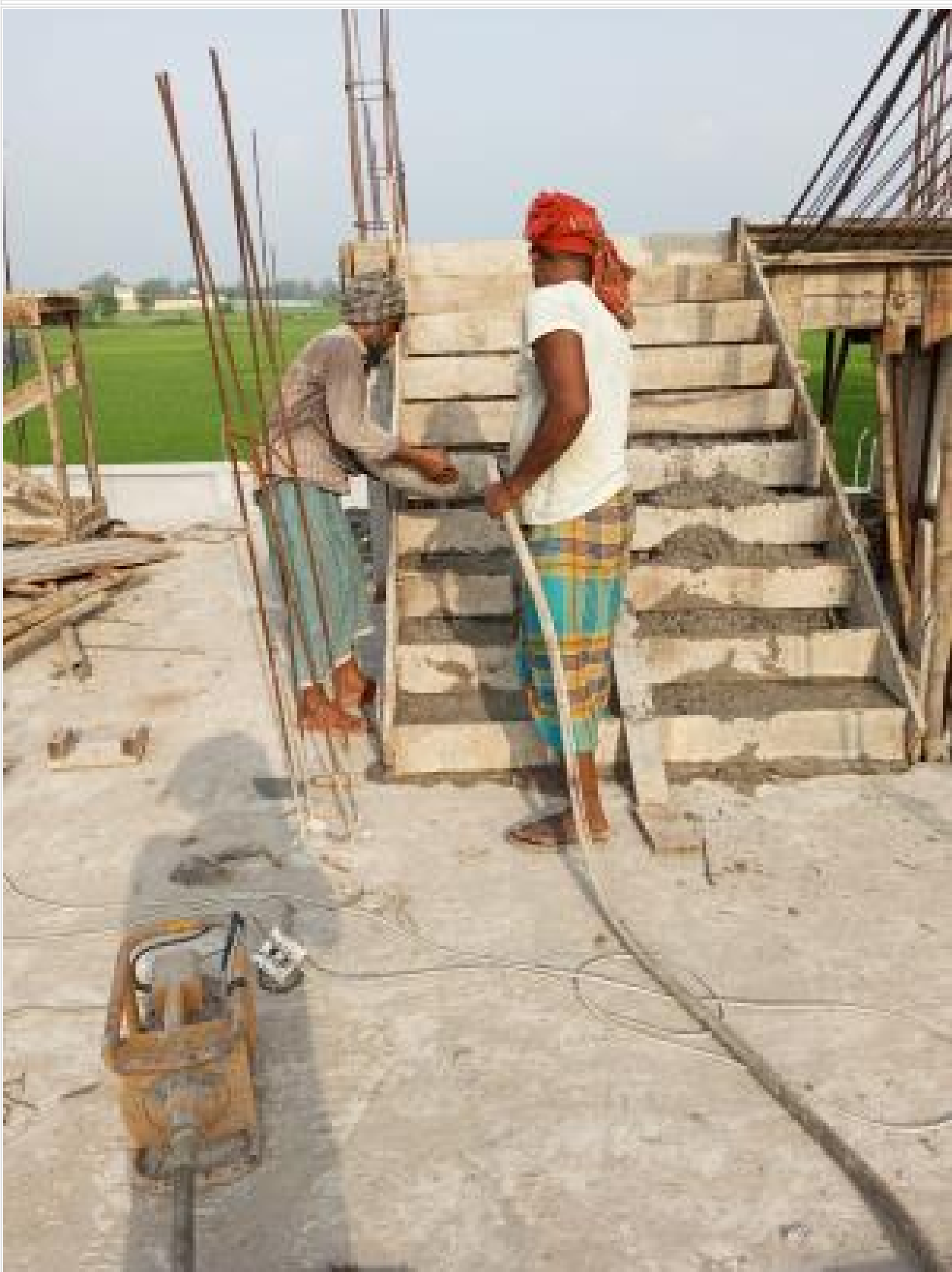
Dorm. Bldg. 1st flight stair casting on 30-08-23
