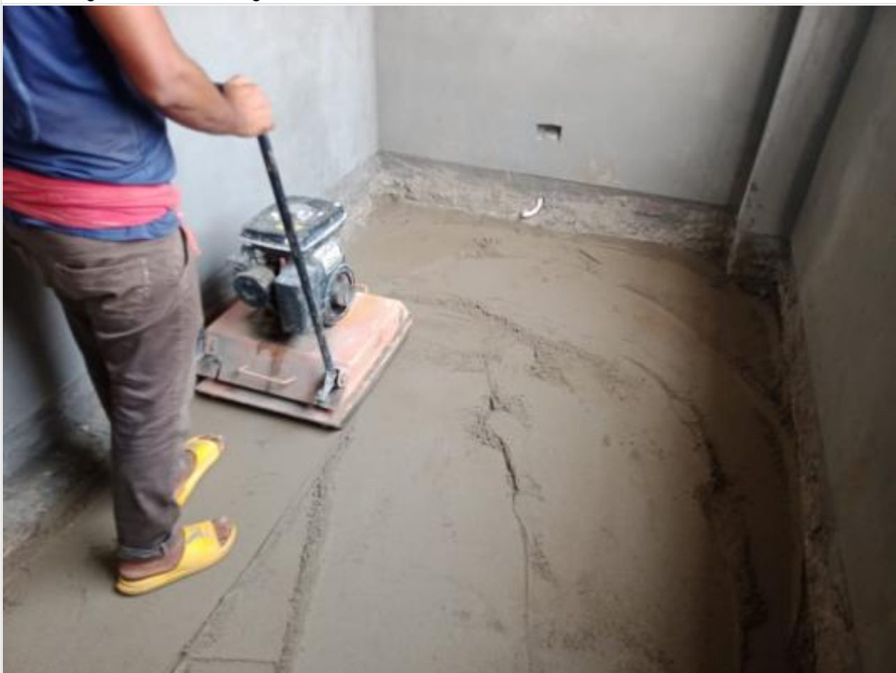
Dorm. Bldg. GF sand khoa cushion on 09-11-23
