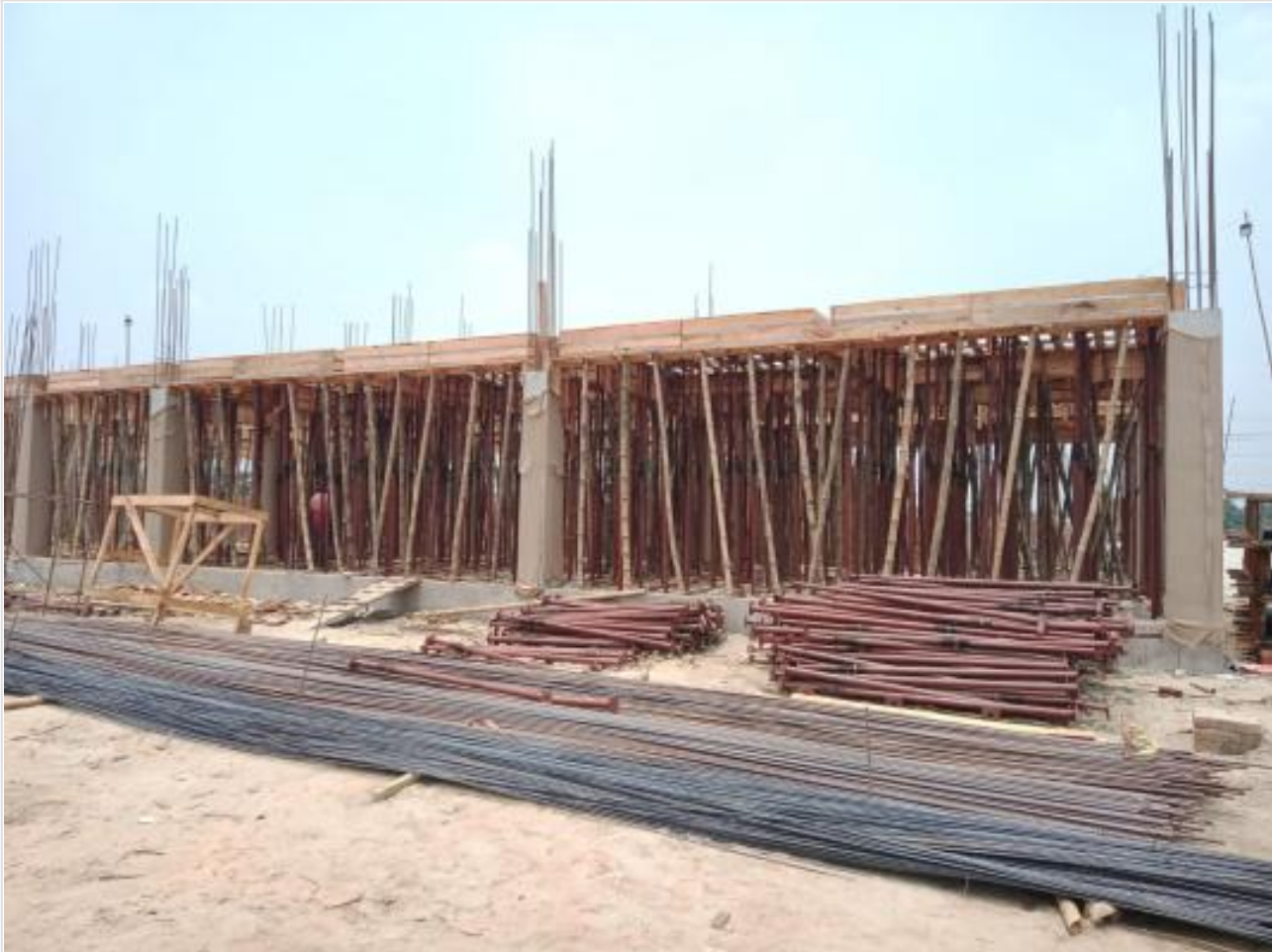
Comp. Bldg. Slab beam shuttering on 10-06-23
