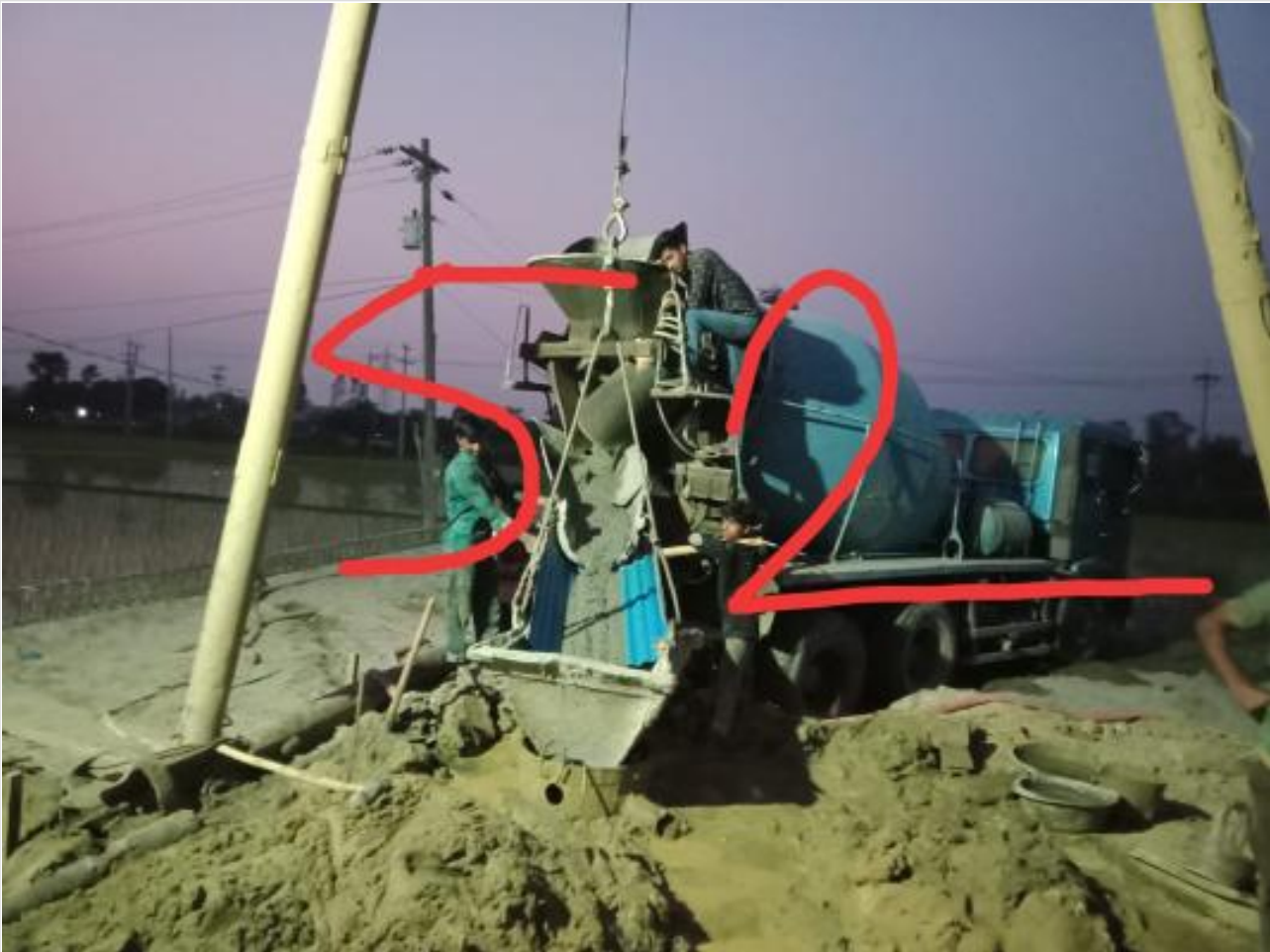
Ready mix concreting of pile on 10-03-23
