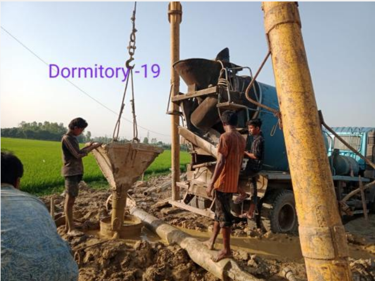
Pile cap bottom cc casting. on 04-04-23
