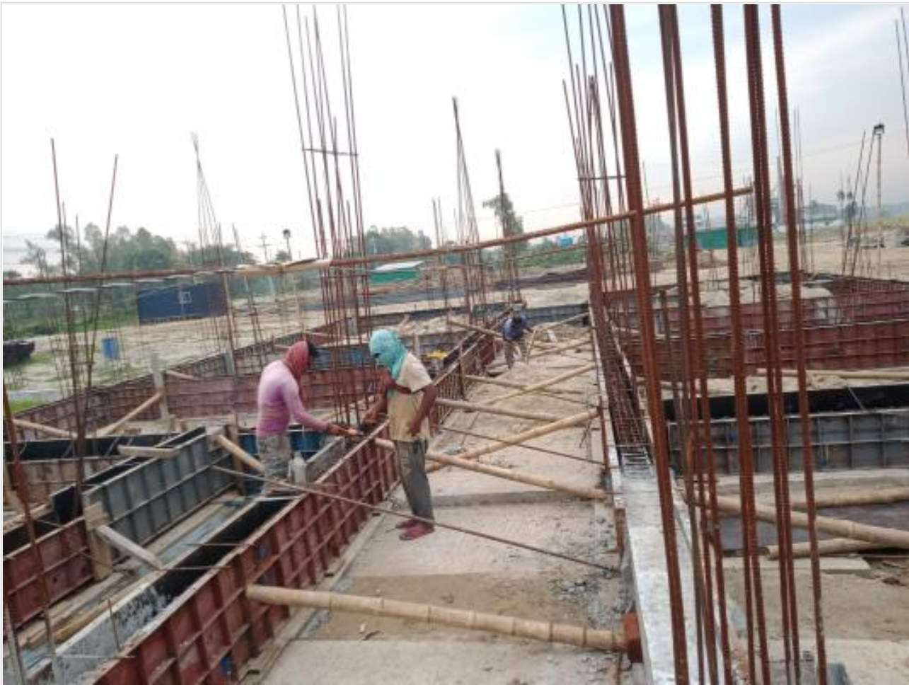
Com Bldg GB Shuttering on 15-05-23
