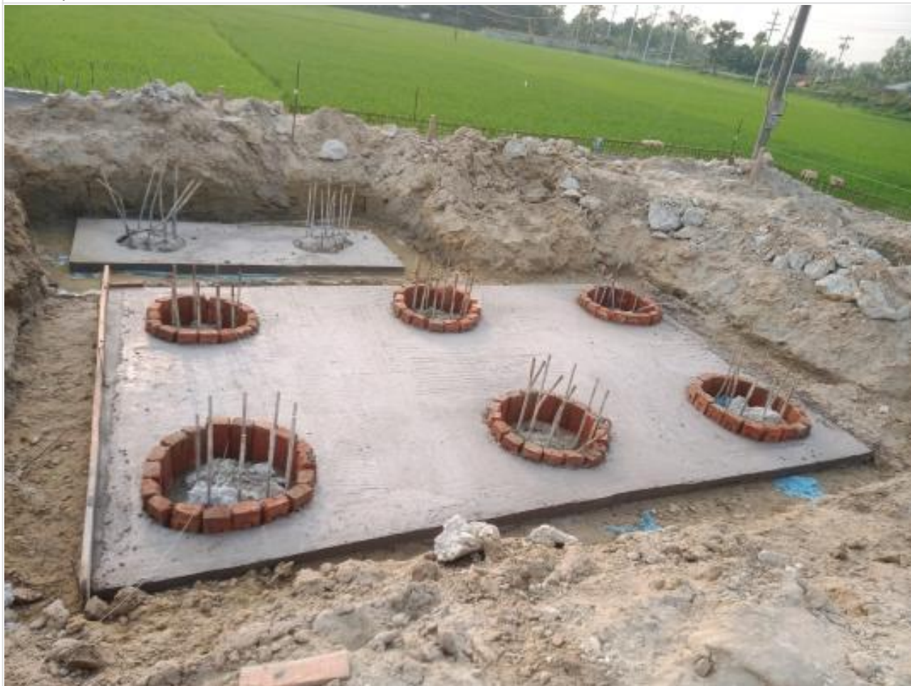
Pile cap bottom cc casting. on 04-04-23
