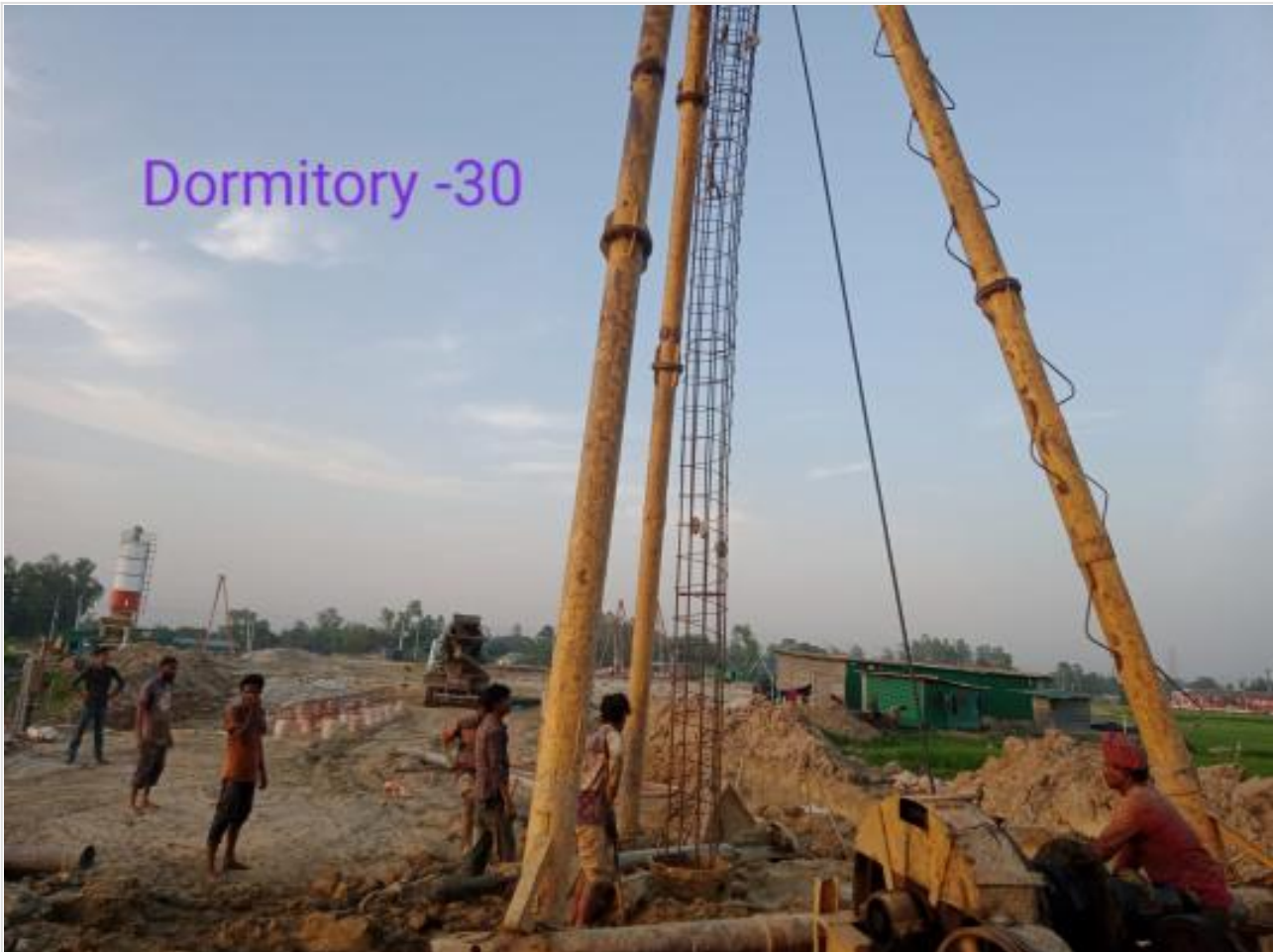
Pile head finishing for test on 07-04-23
