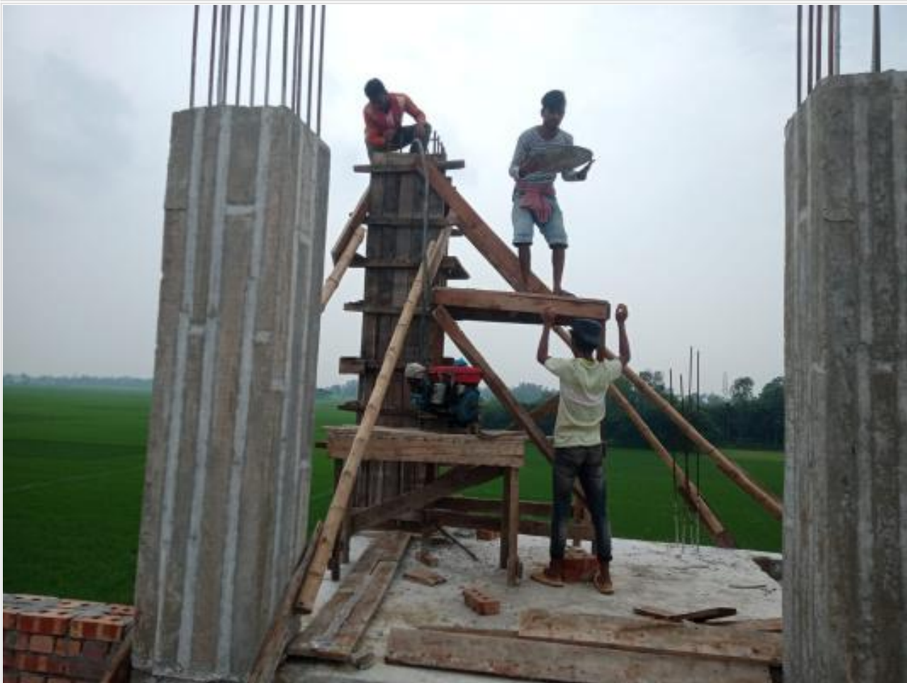
Comp. Bldg Column casting on 27-08-23
