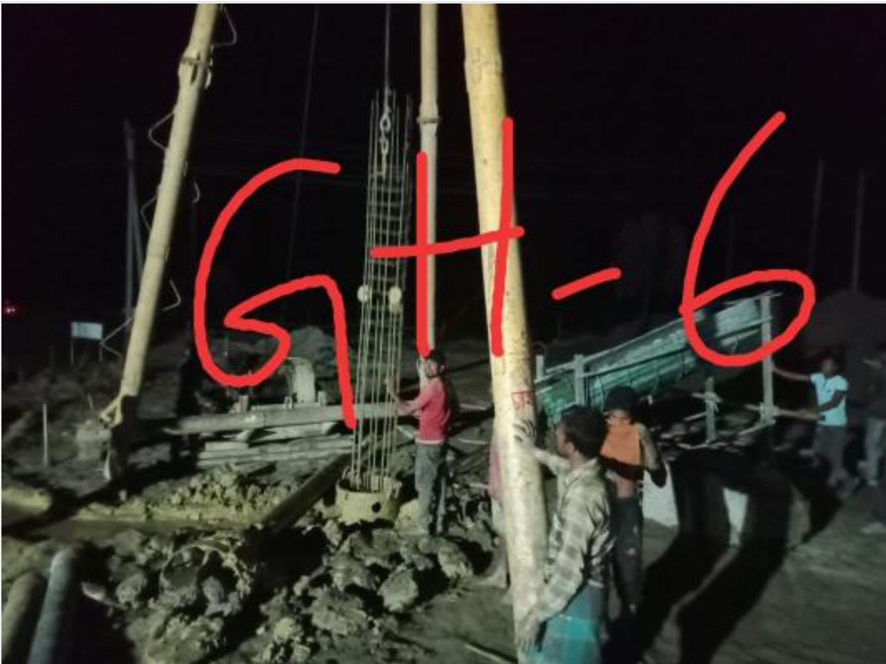
Guard House pile concreting by RMC on 19-03-23
