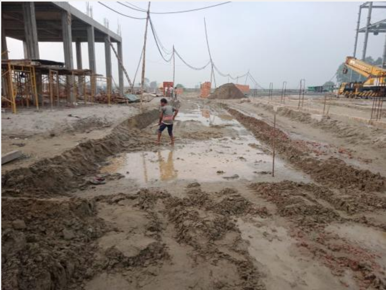
Road-Excavation-box cutting on 16-08-23
