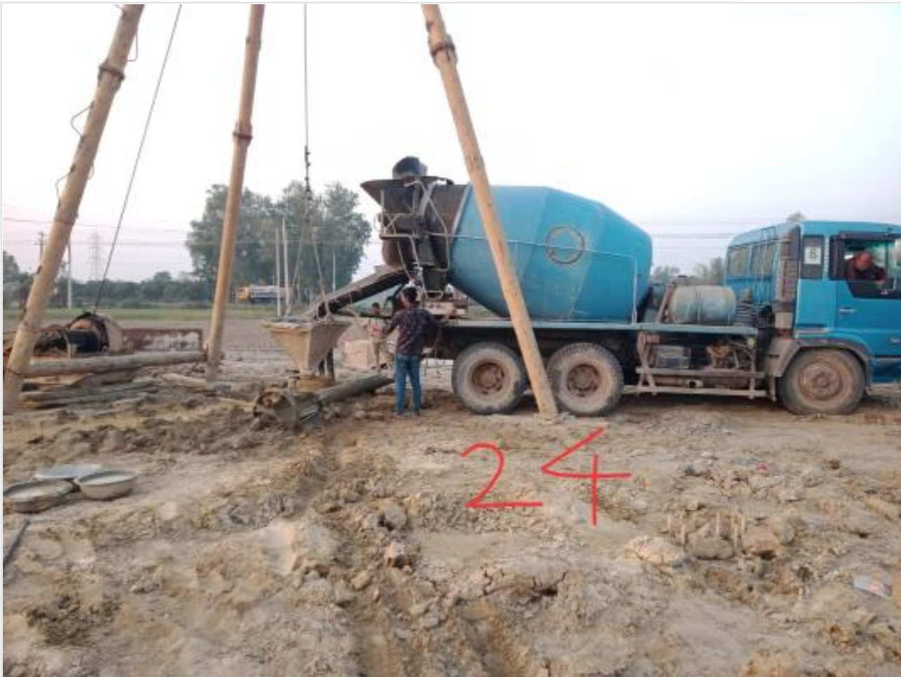
Ready mix concreting of pile on 24-02-23
