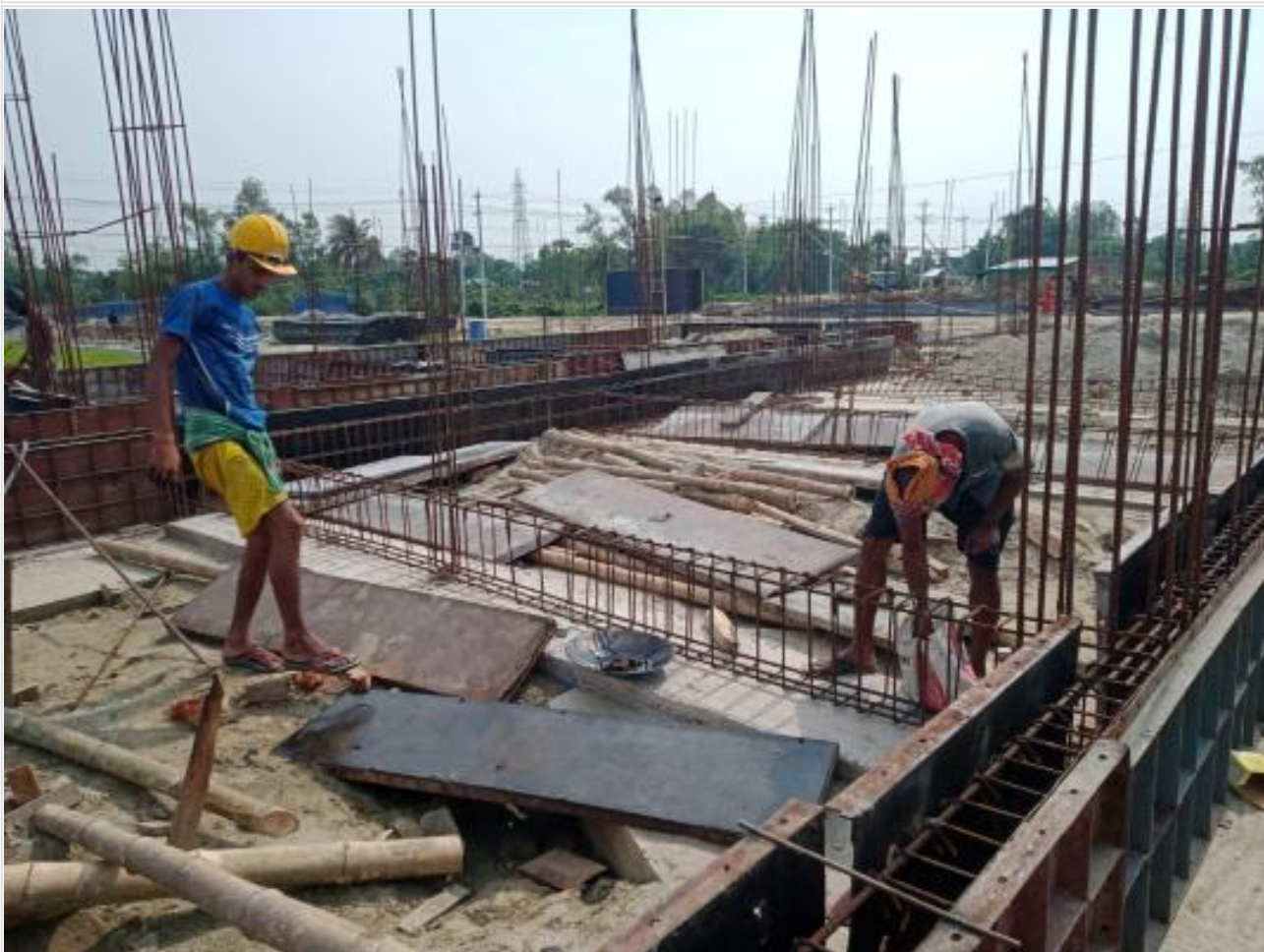
Comp. Bldg. GB Shuttering work on 14-05-23
