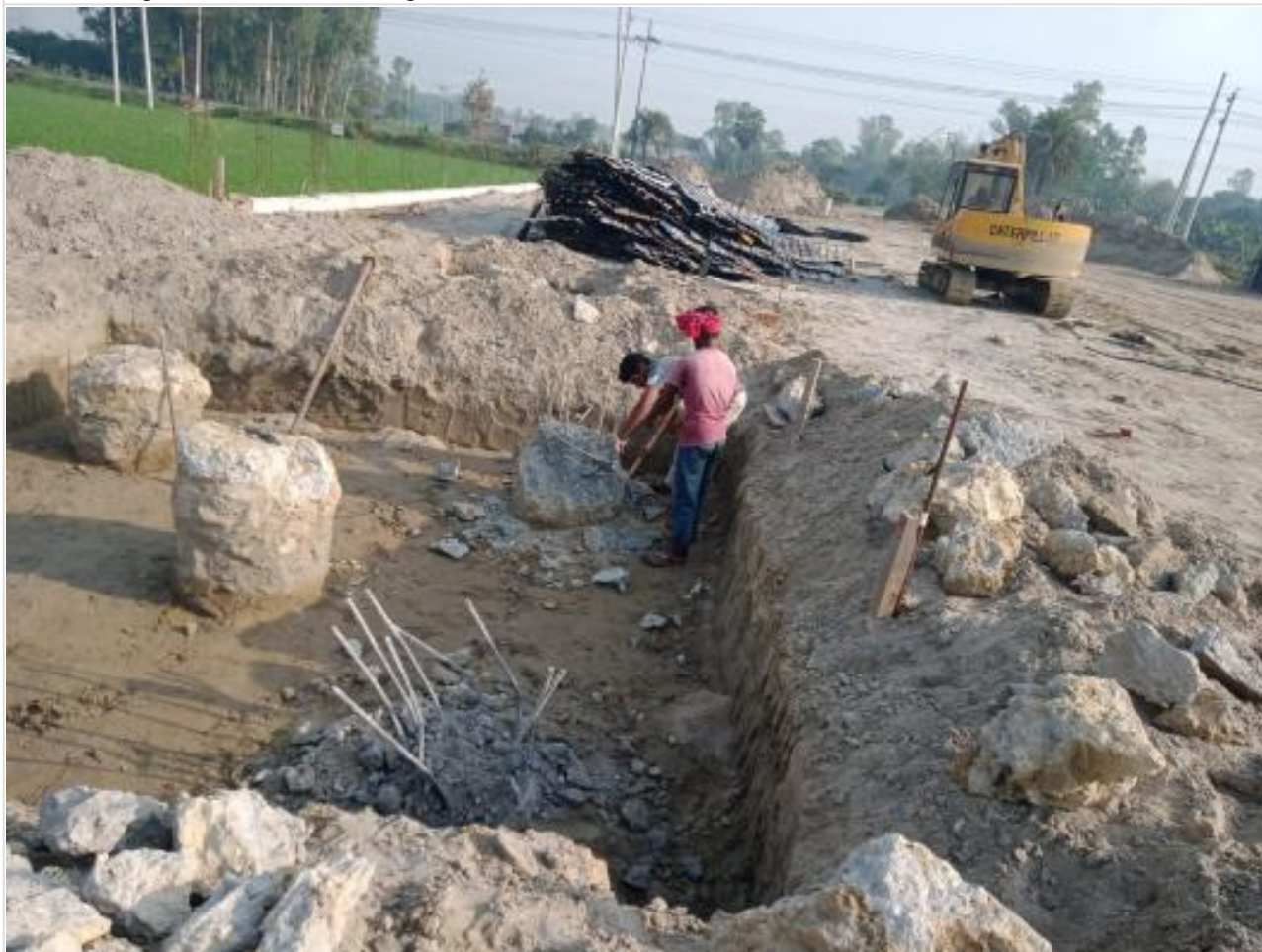
Pile head breaking on 28-03-23
