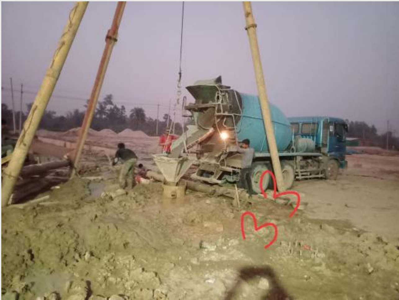
Ready mix concreting of pile on 27-02-23
