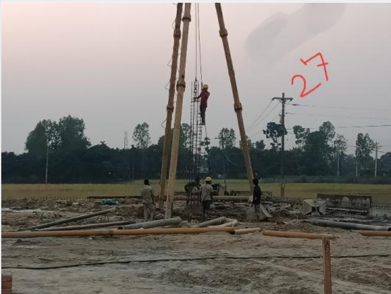
Com. Bldg. 27th pile boring on 25-02-23
