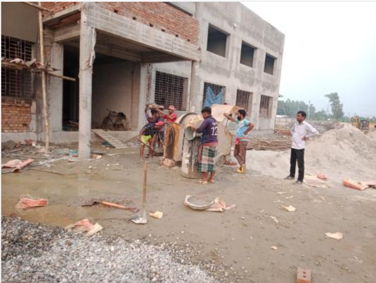
Comp. Bldg. GF casting on 16-10-23
