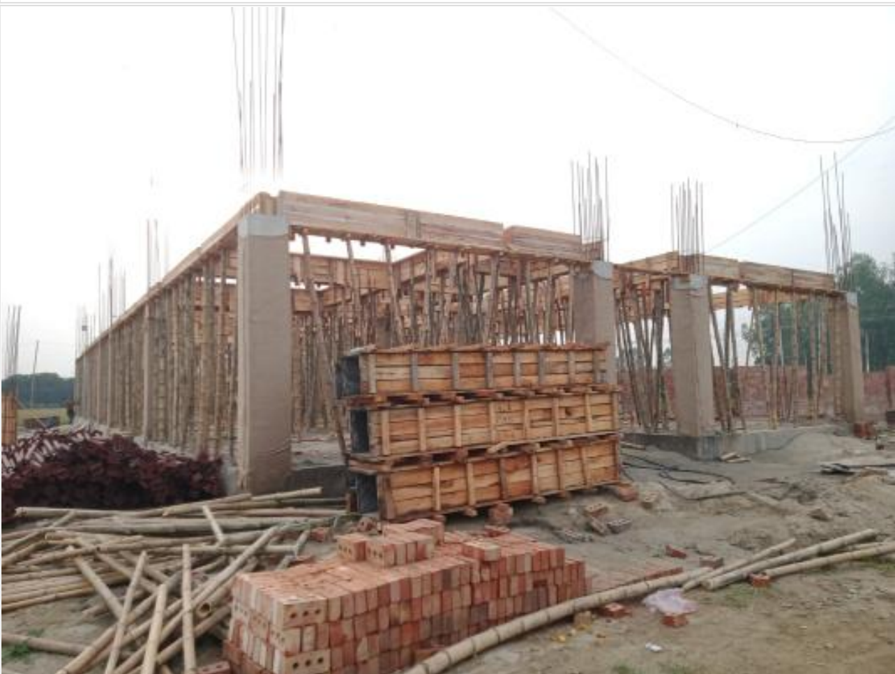
Comp. Bldg. Slab beam shuttering on 07-06-23
