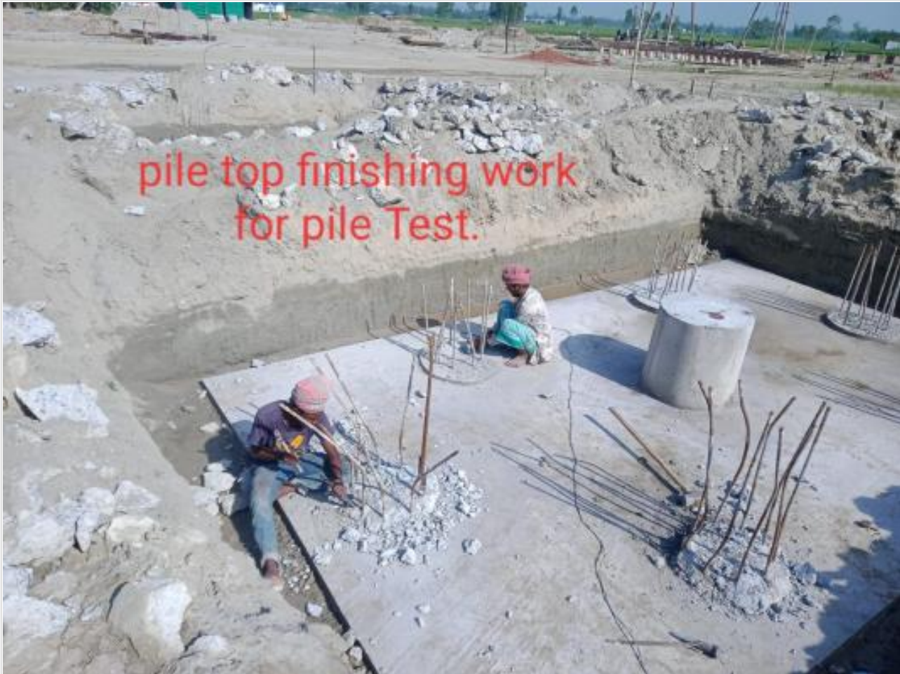
Pile head finishing for test on 07-04-23
