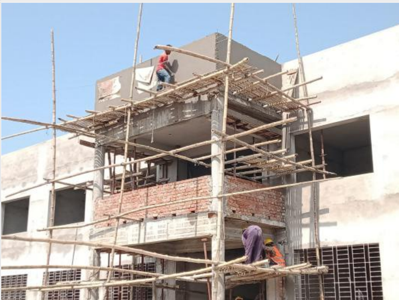
Comp. Building-Outside Plastering on 20-10-23
