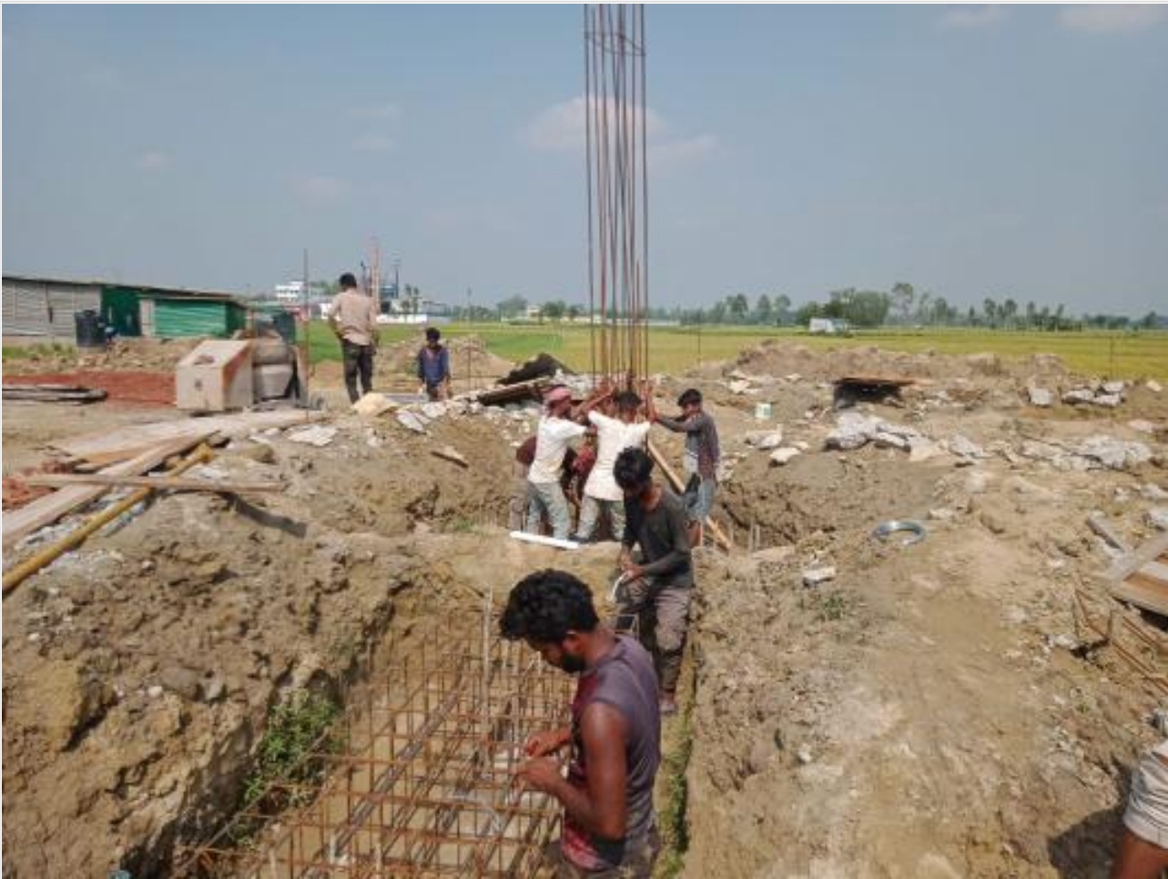
Dorm. Bldg. Pile cap rebar binding on 24-05-23
