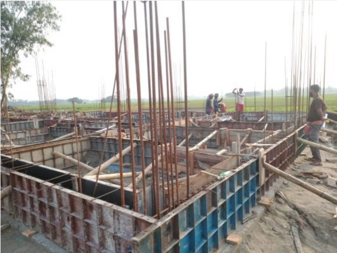
Dorm. Bldg. GB shuttering on 12-06-23
