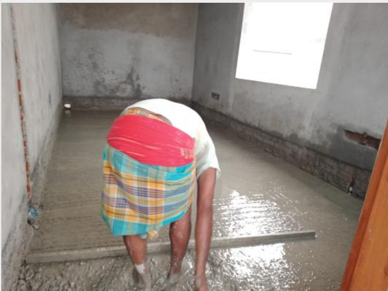
Gate House floor casting on 01-09-23
