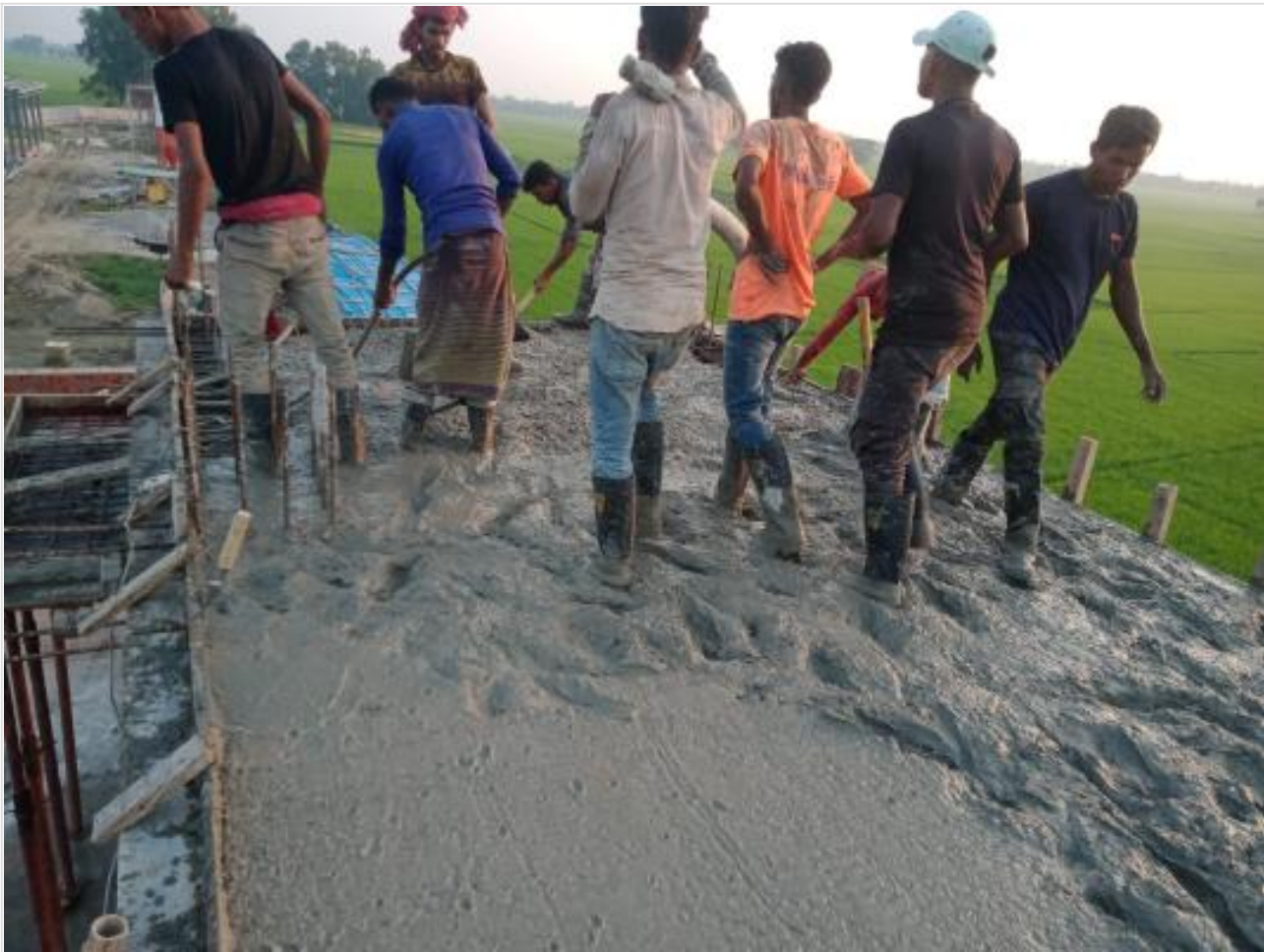
Comp. Bldg. Roof top concreting work on 16-09-23
