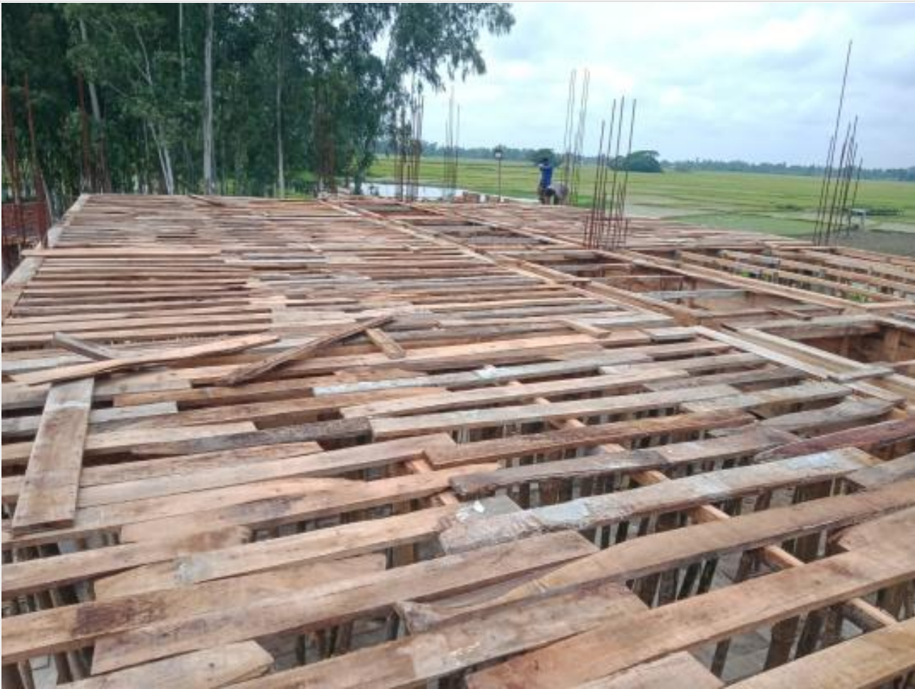
Dorm. Bldg shuttering work on 28-07-23
