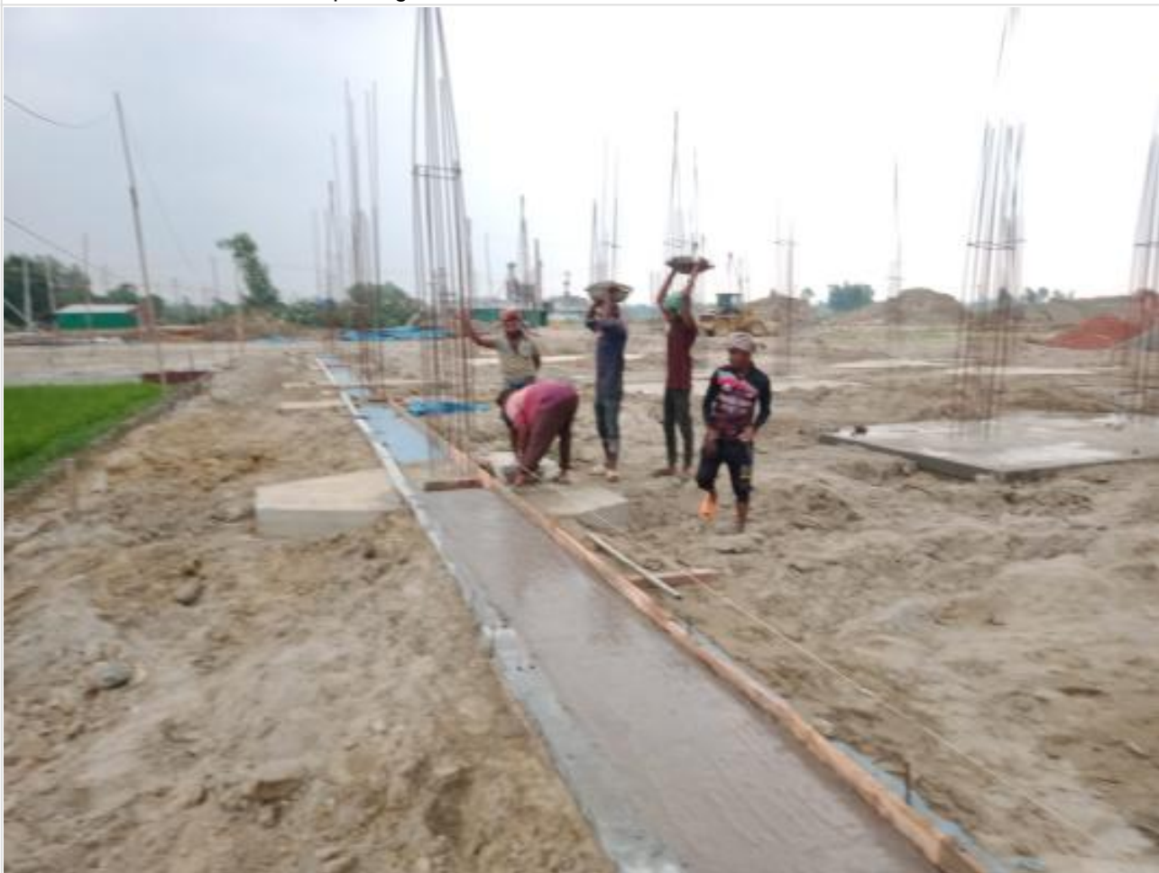
Comp. Bldg. C.C concreting on 29-04-23
