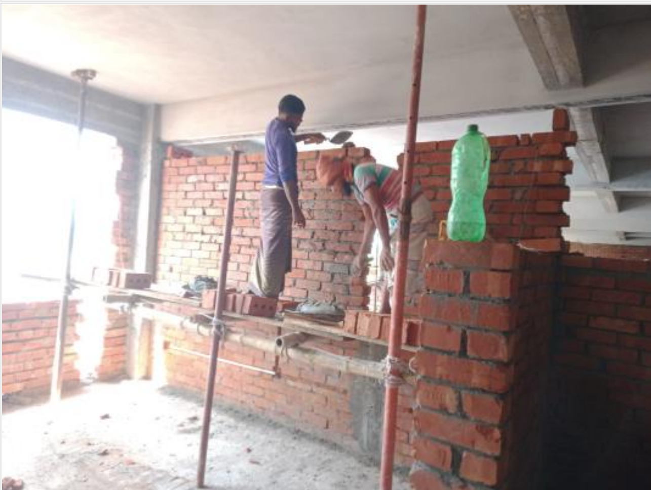
Comp. Bldg. 2nd Floor work on 10-09-23
