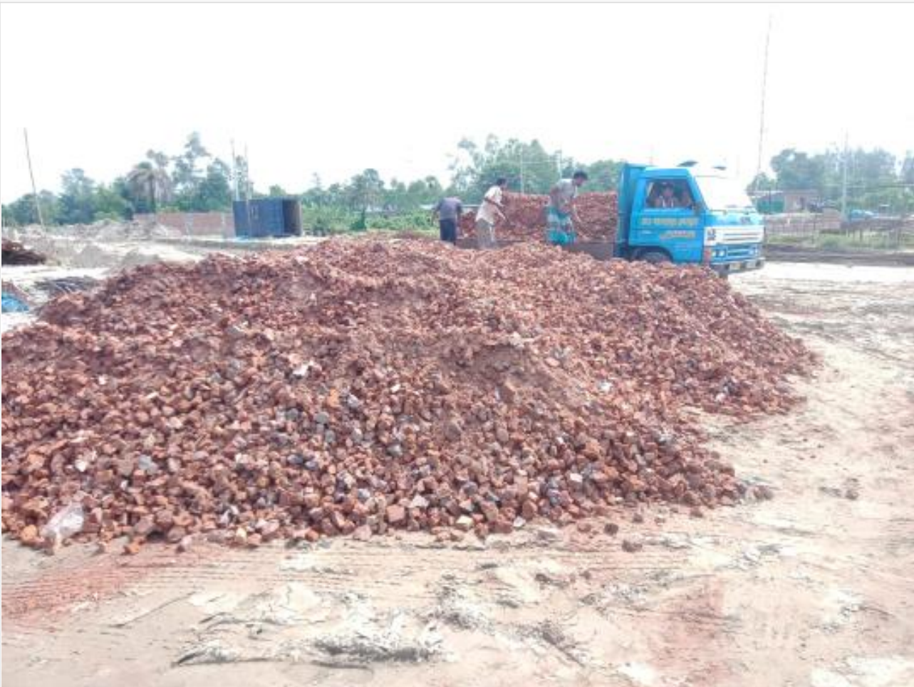
Materials arrive at site for road on 19-07-23
