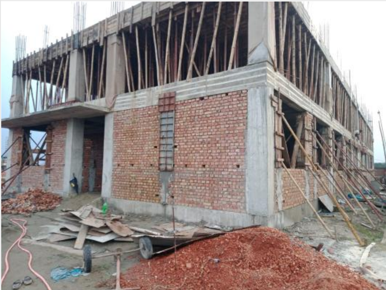
Comp.Bldg.GF Brick work on 09-08-23
