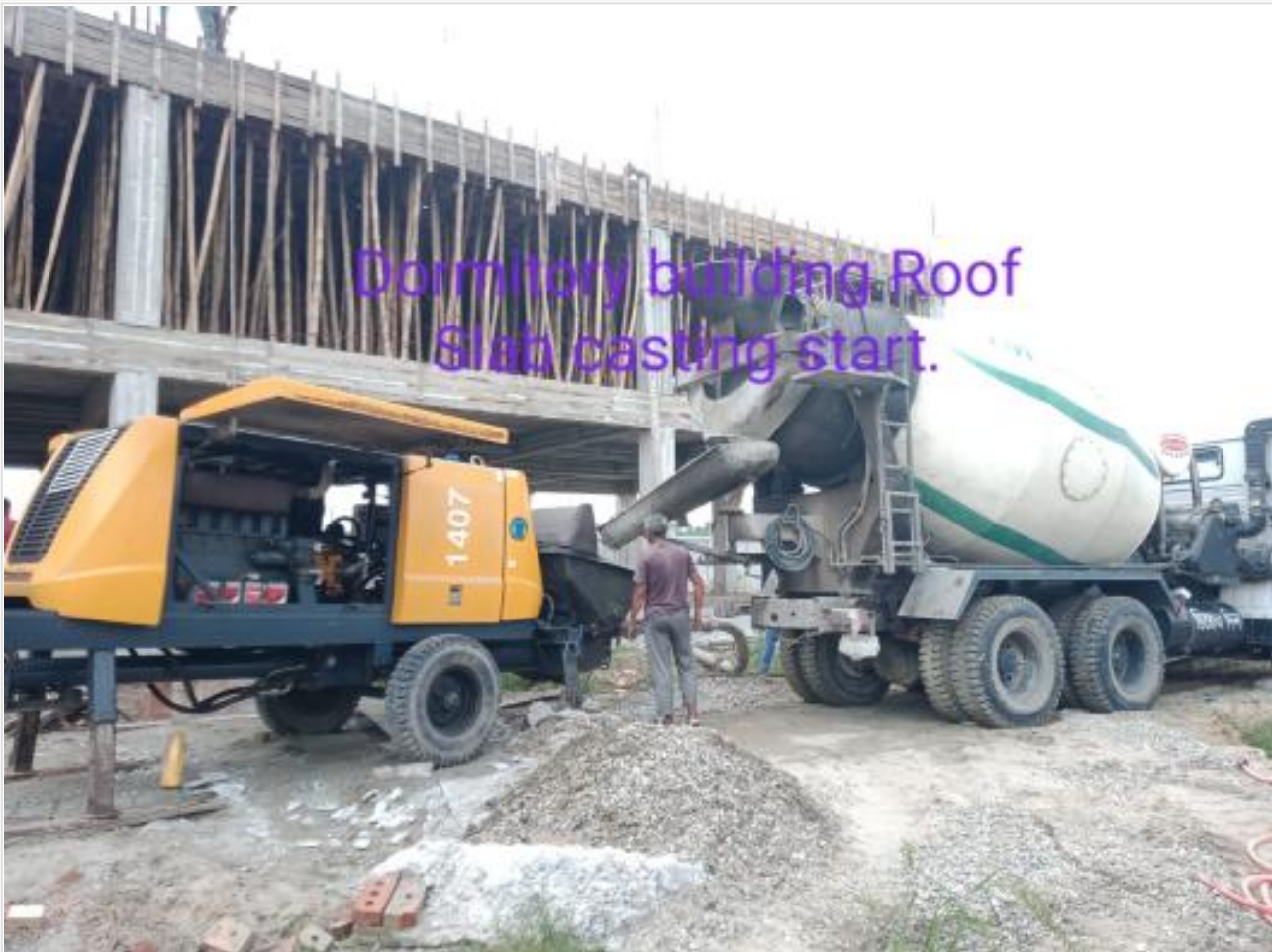
Dorm. Bldg. 2nd floor concreting work on 16-09-23
