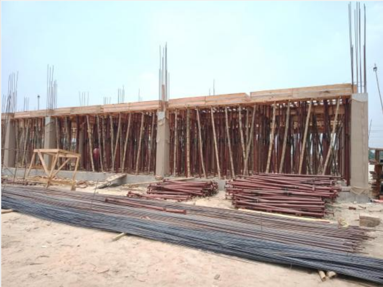
Comp. Bldg. Slab beam shuttering on 10-06-23
