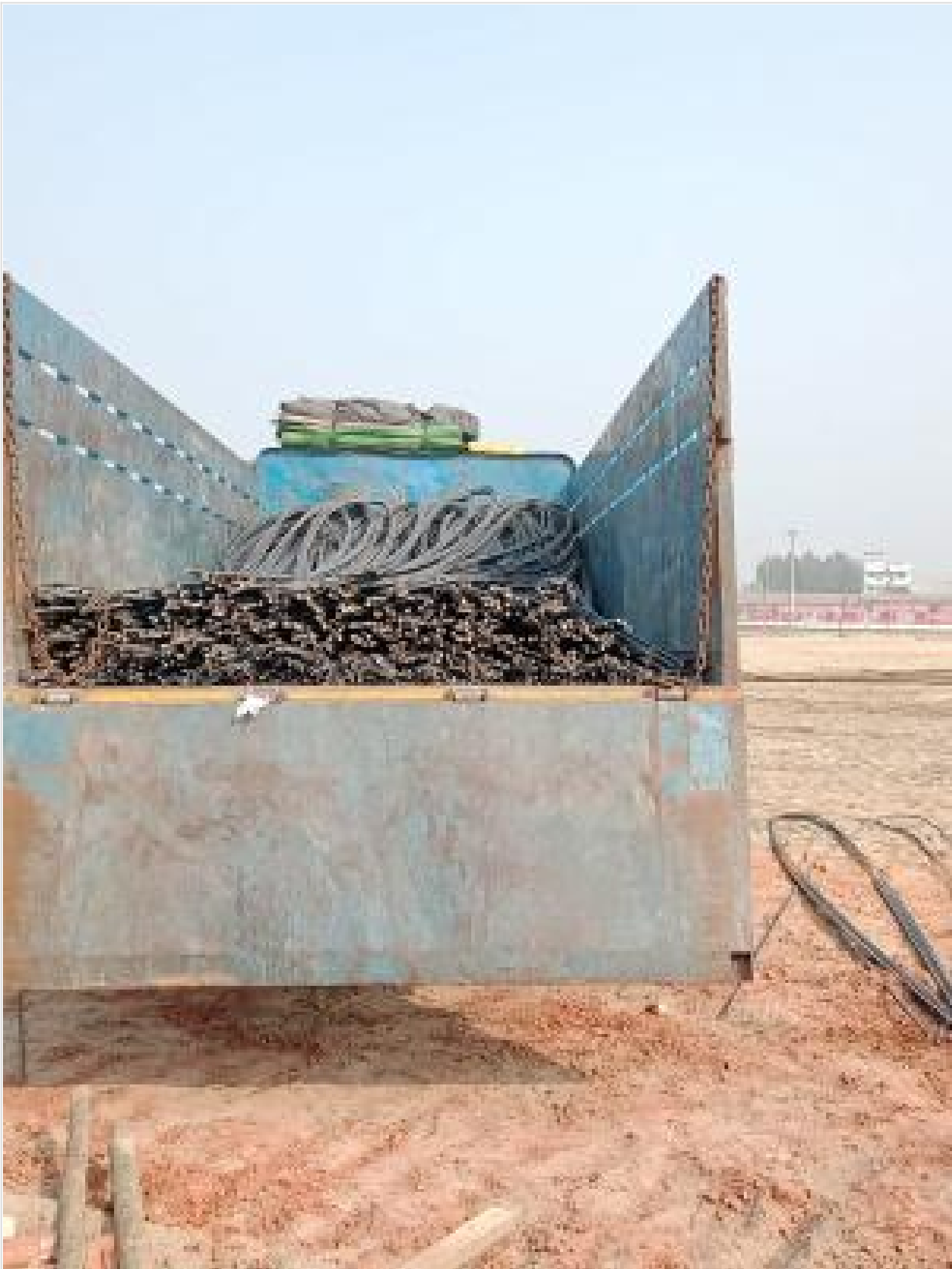
Re-bar mobilized on 21-01-23
