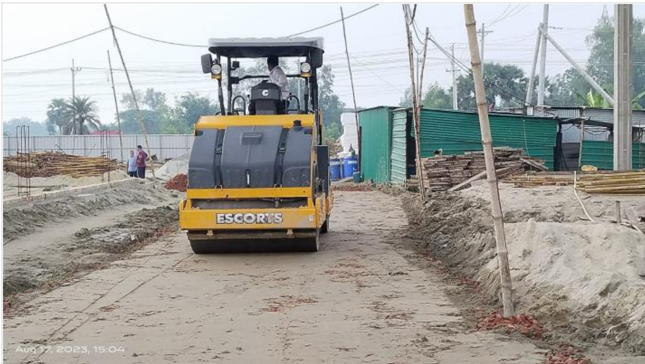
Sub-base Compaction on 17-08-23
