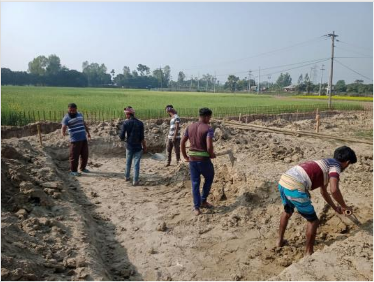
Exaction for Pile mud tank on 02-02-23
