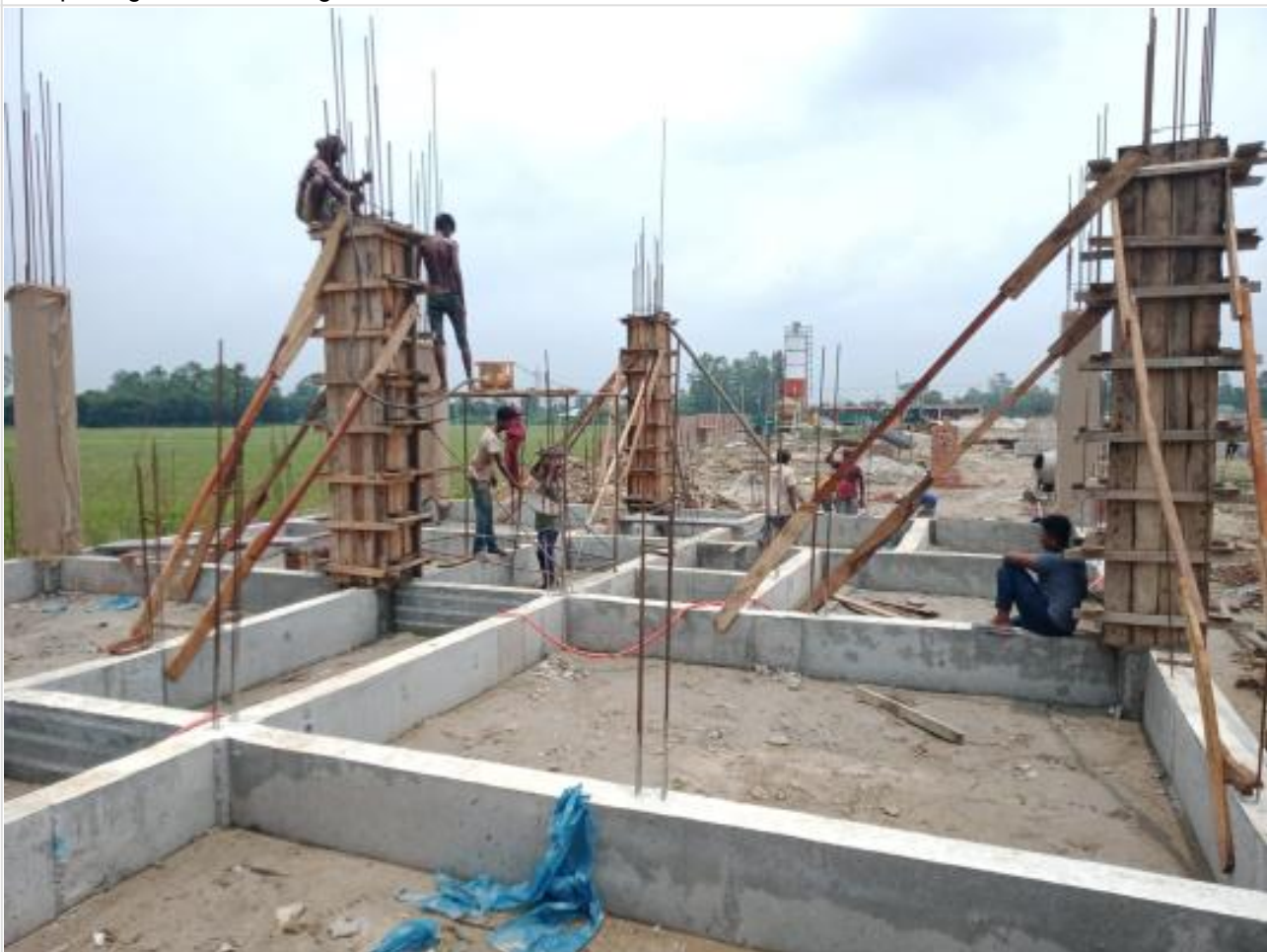
Dorm. Bldg. Column casting on 20-06-23
