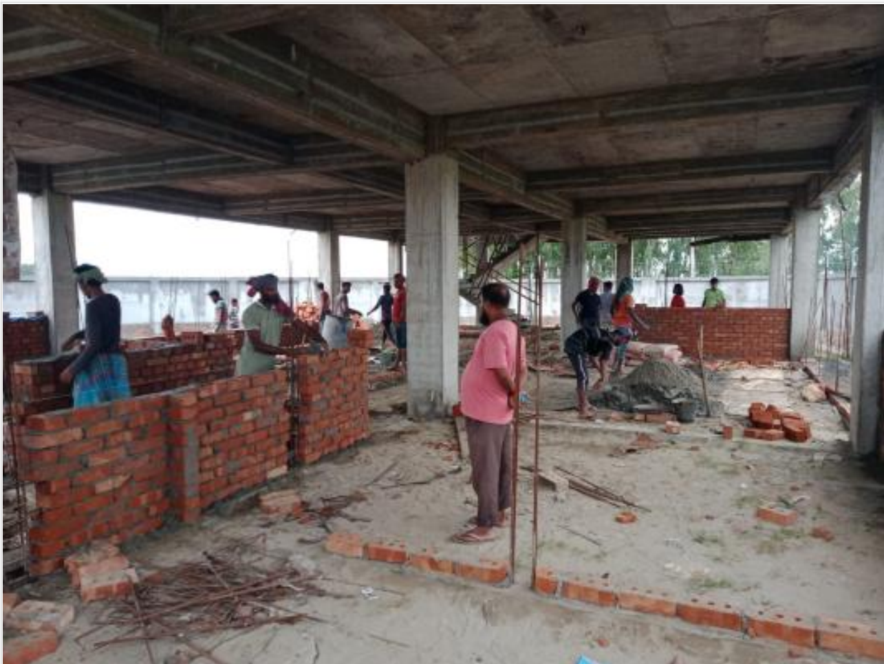
Dorm. Bldg GF Brick work on 22-09-23
