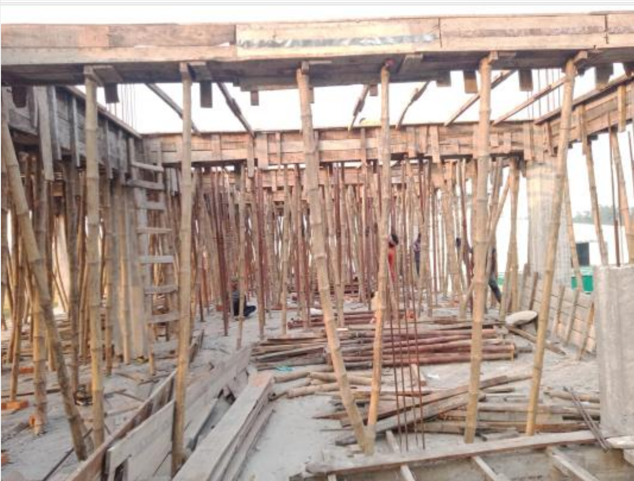
Dorm. Bldg. 3rd floor slab shuttering on 08-11-23
