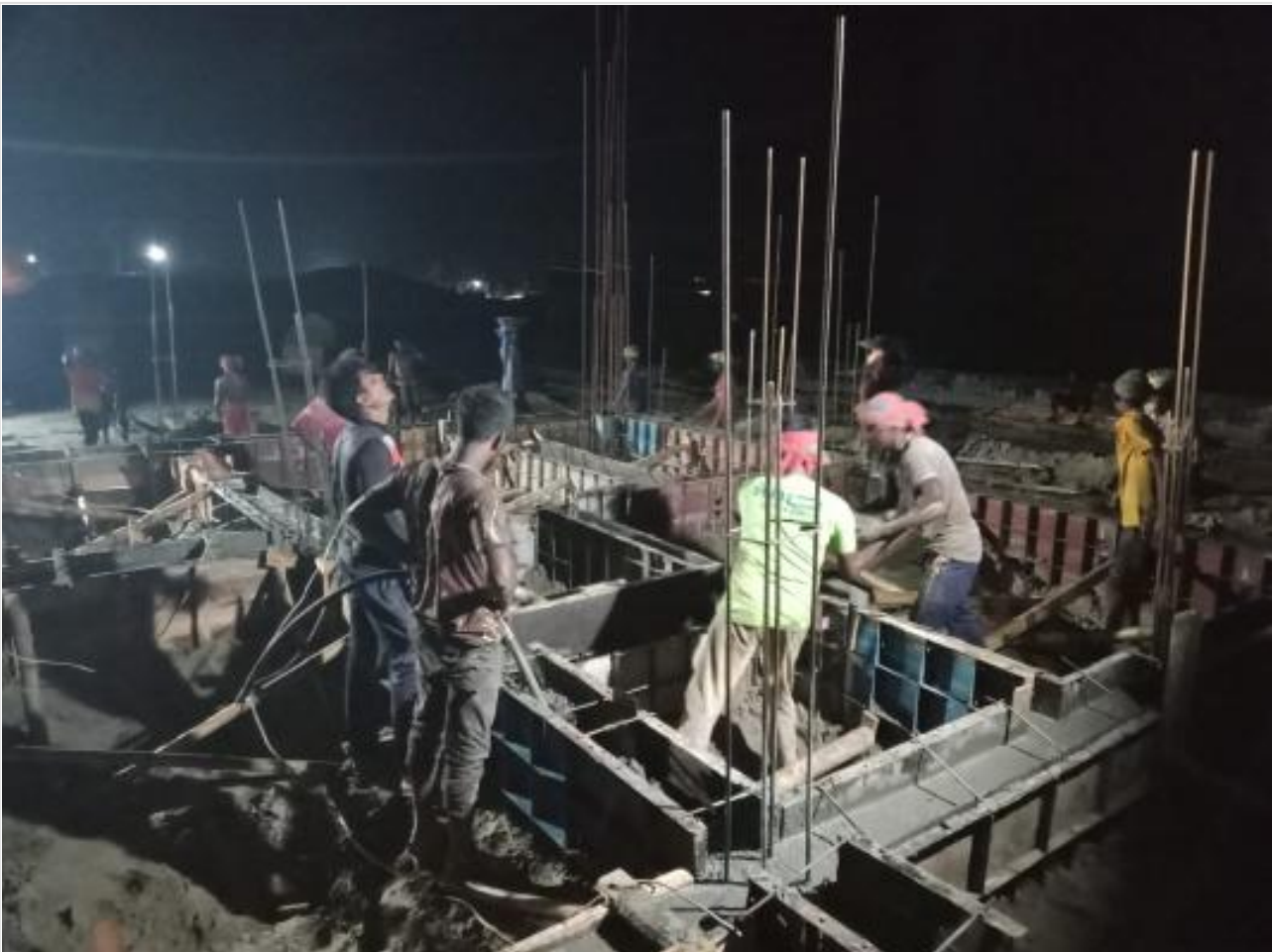
Dorm. Bldg. GB shuttering on 12-06-23
