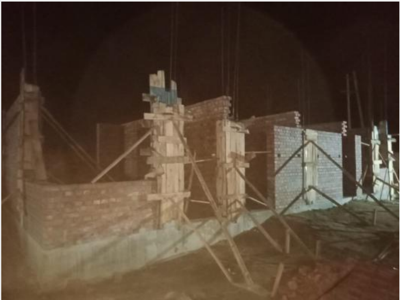
Gate House column casting on 18-06-23
