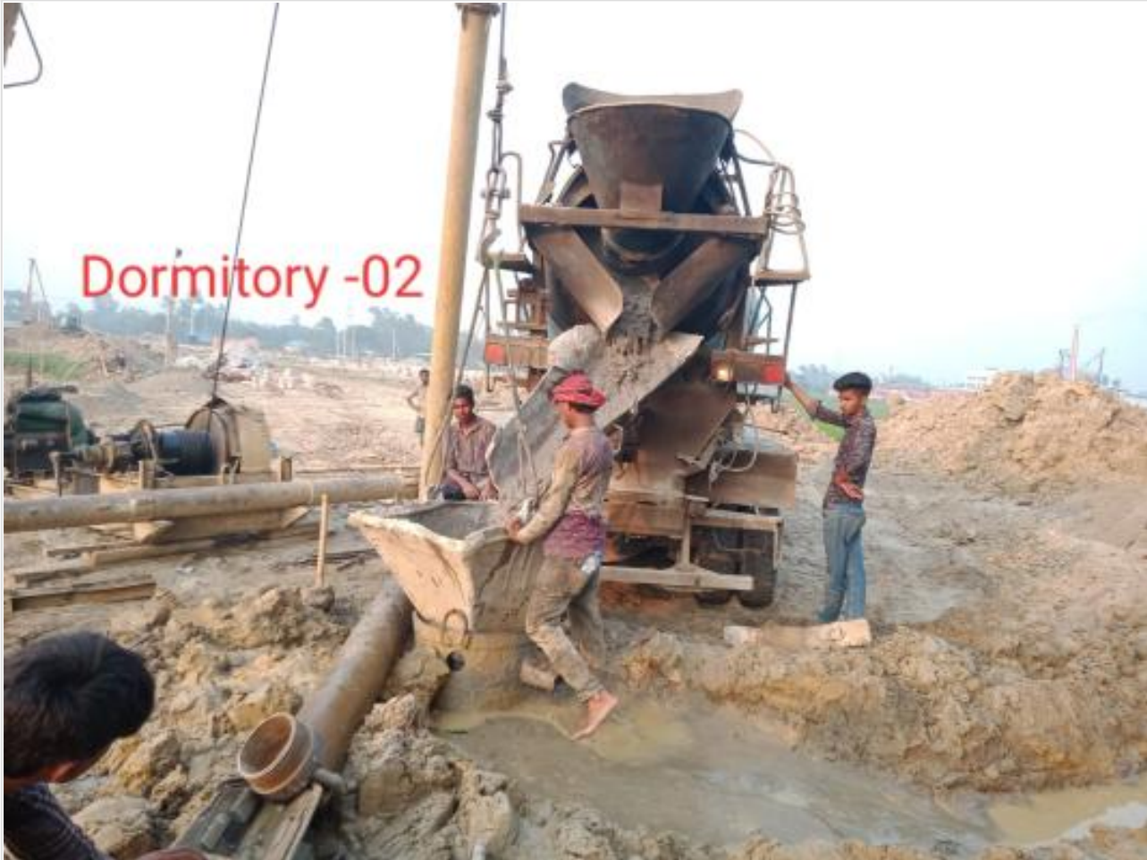
Ready mix concreting of pile on 25-03-23
