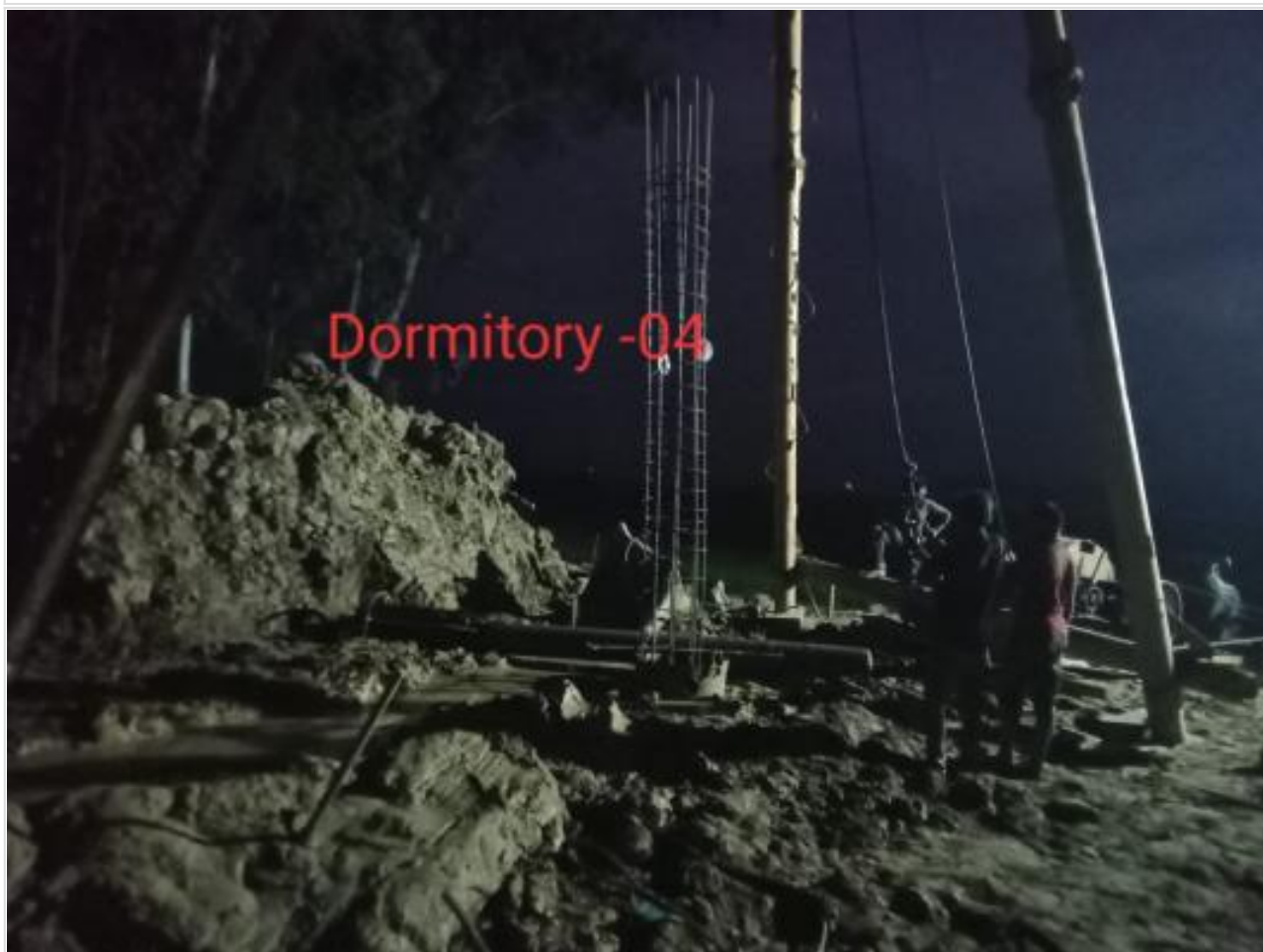
Ready mix concreting of pile on 25-03-23
