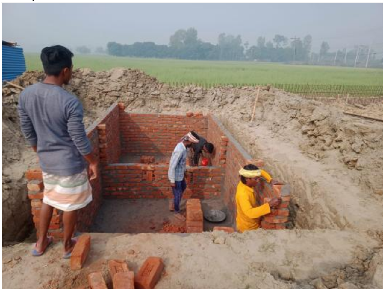
Mud Tank making on 06-02-23
