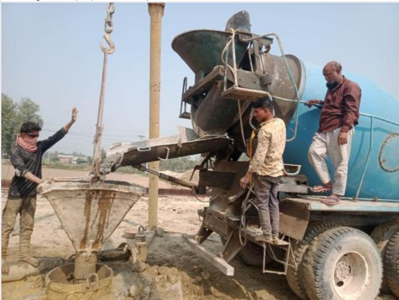
Ready mix concreting of pile on 15-02-23
