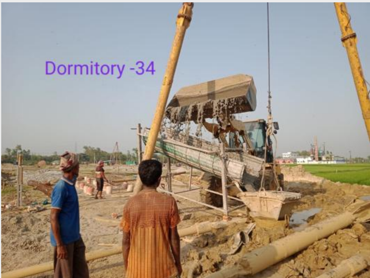
Dorm. Bldg. 32nd pile concreting on 09-04-23
