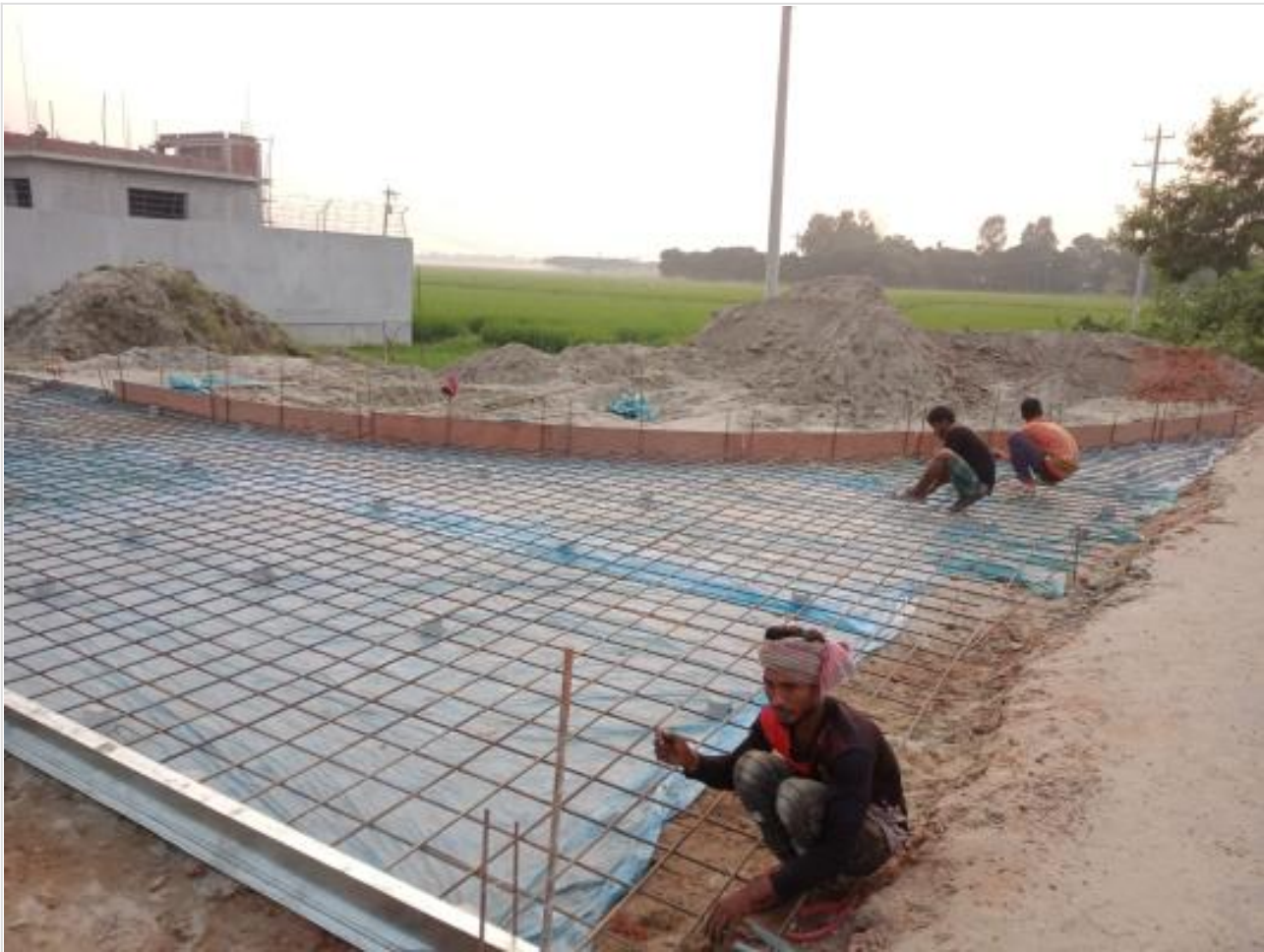
Road work on 15-10-23
