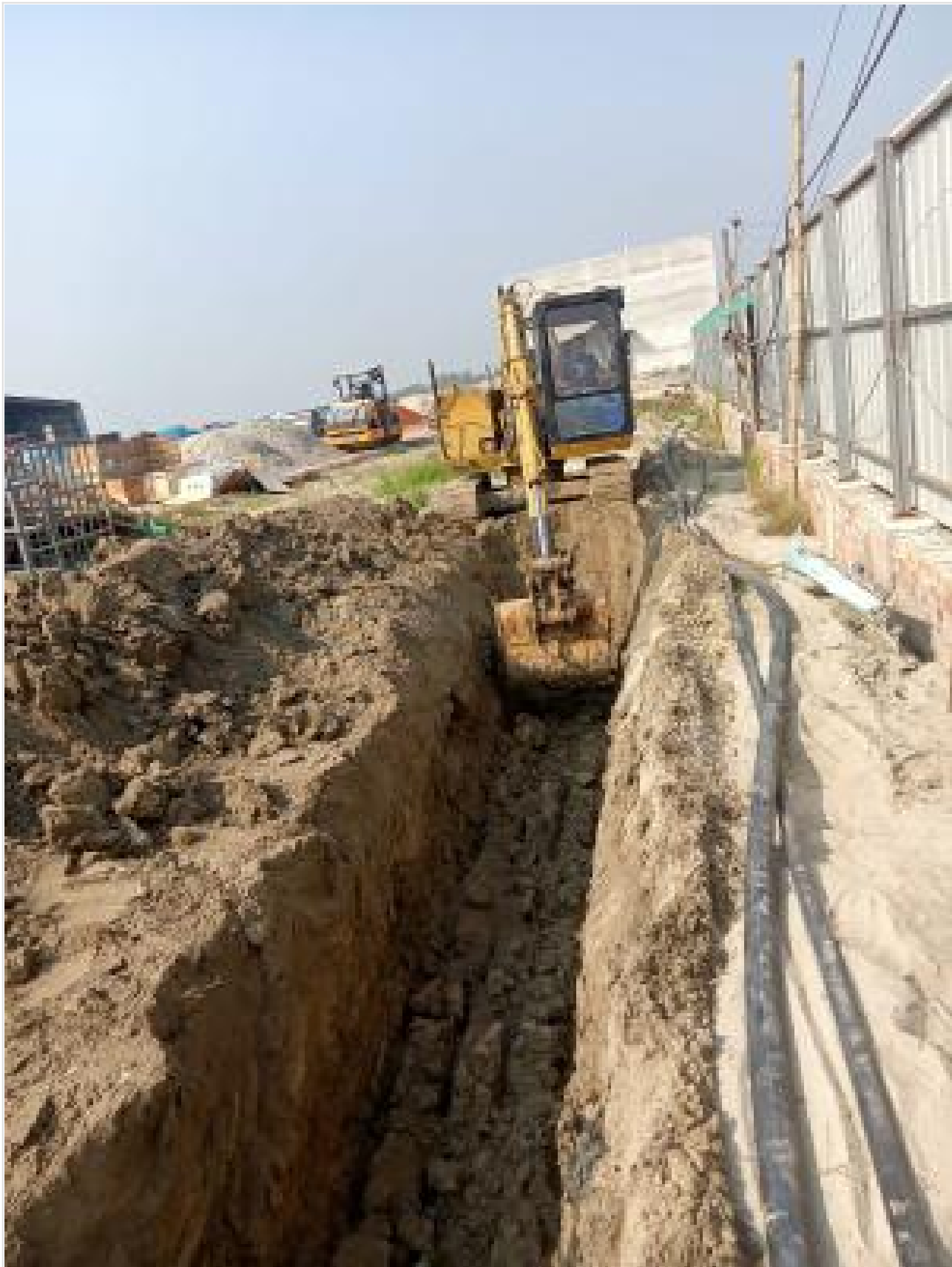
Power cable laying work on 03-11-23
