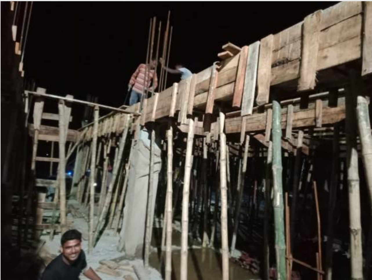
Comp. Bldg. 2nd floor Slab beam shutteri on 17-07-23
