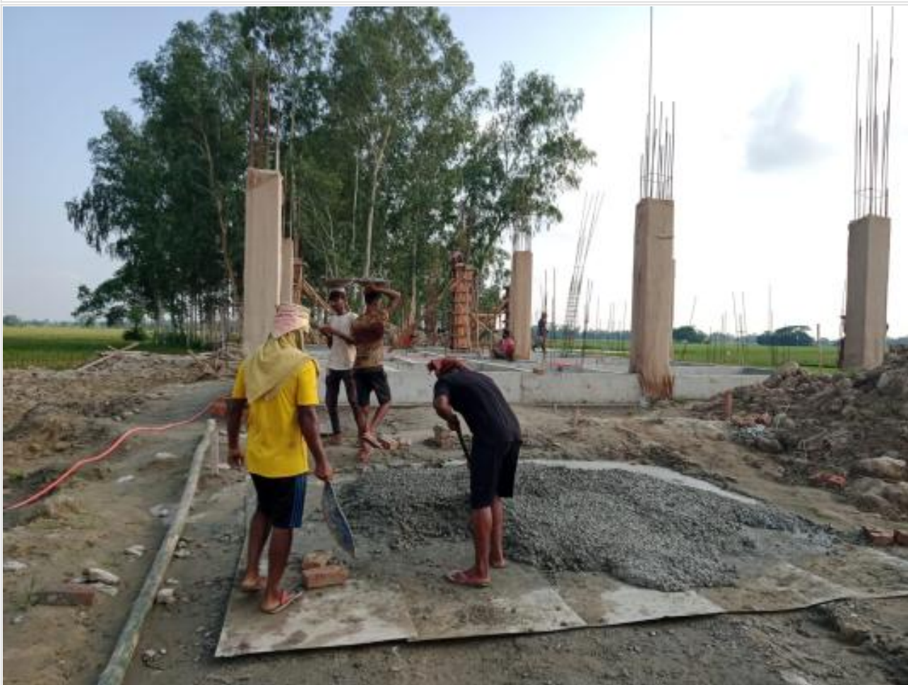
Dorm. Bldg. Column Casting on 23-06-23
