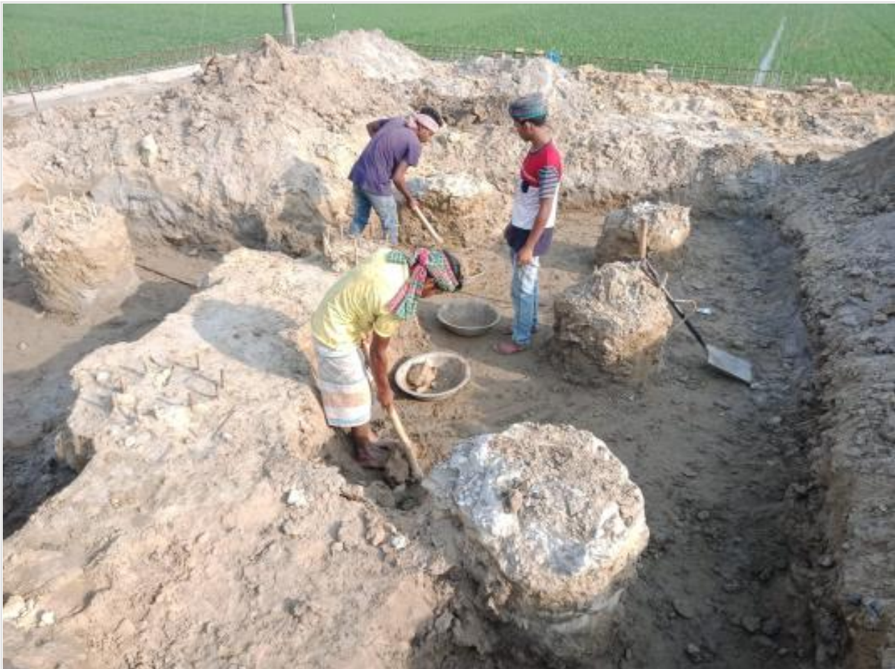
Pile cap earth cutting on 27-03-23
