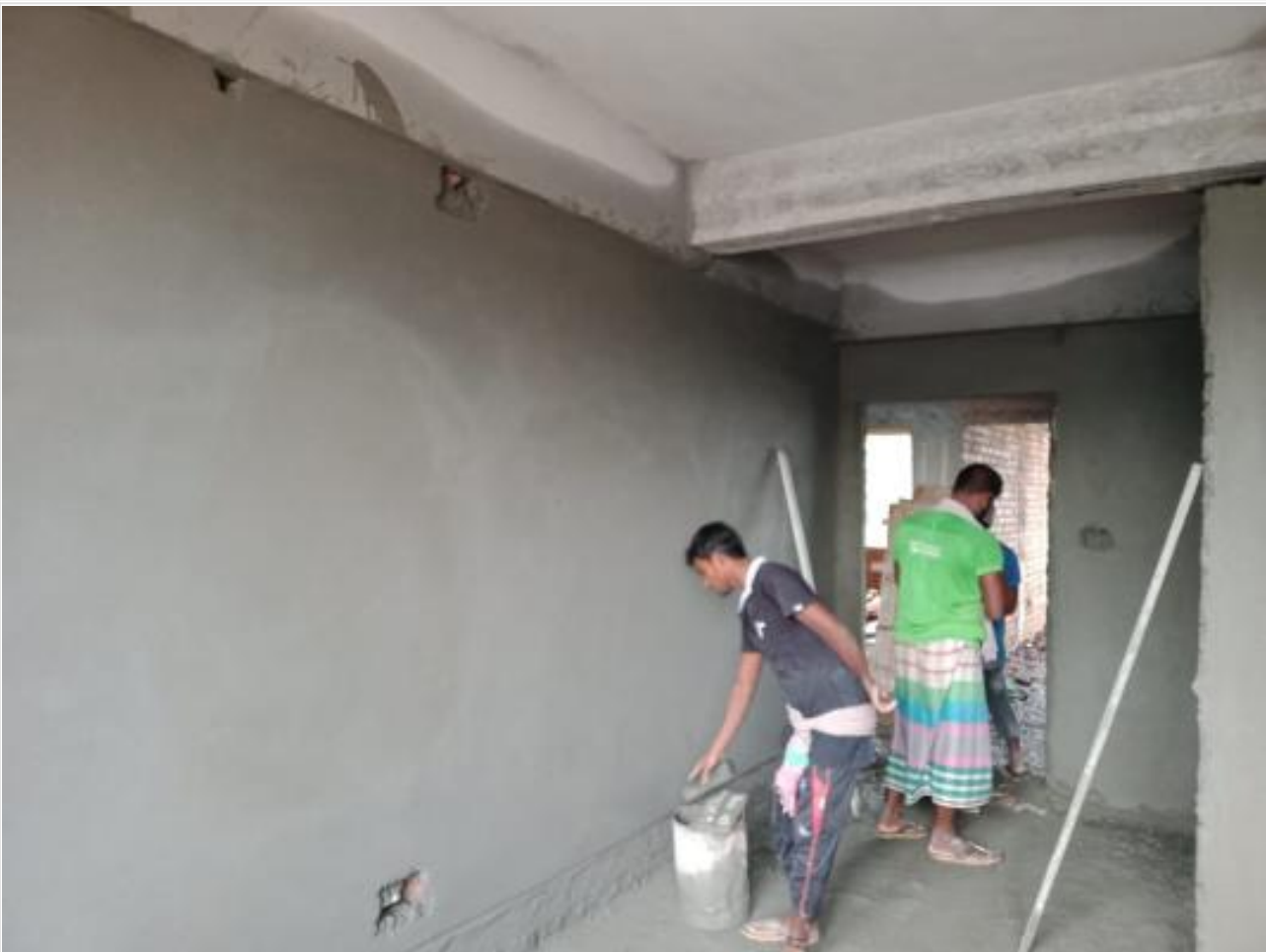
Comp. Bldg. Plaster work on 20-09-23
