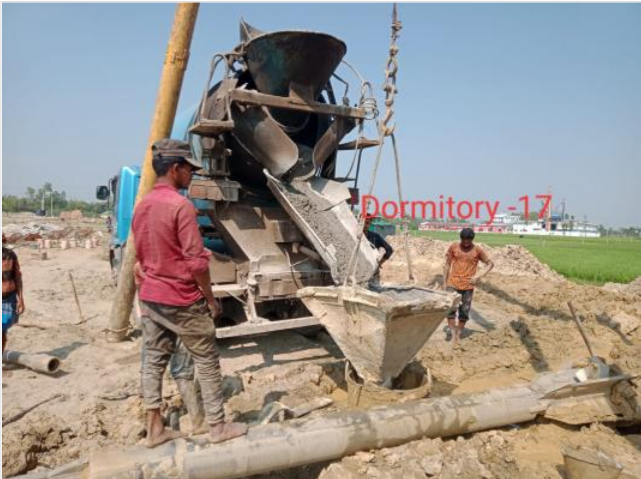
Ready mix concreting of pile on 02-04-23
