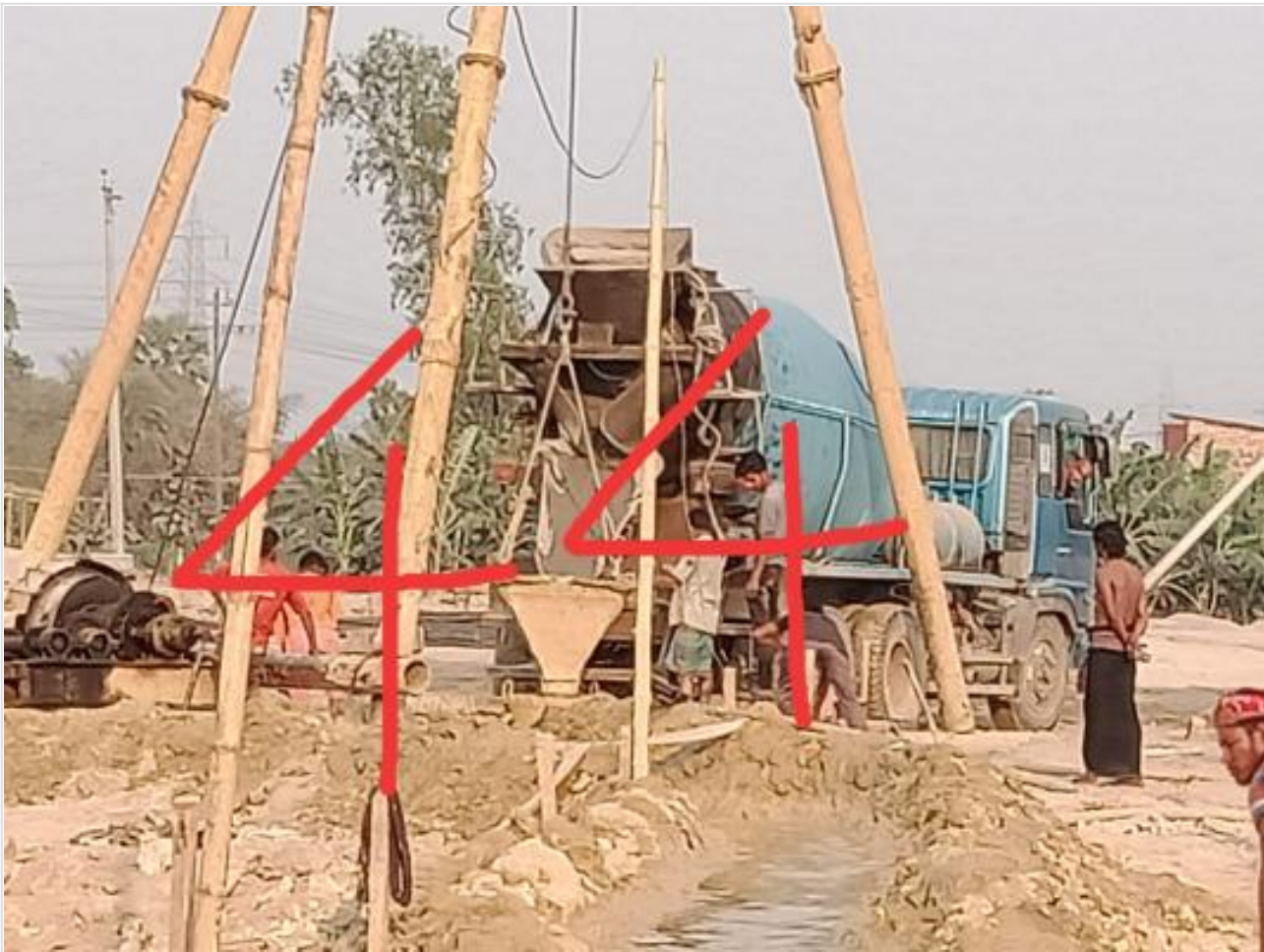
Ready mix concreting of pile on 05-03-23
