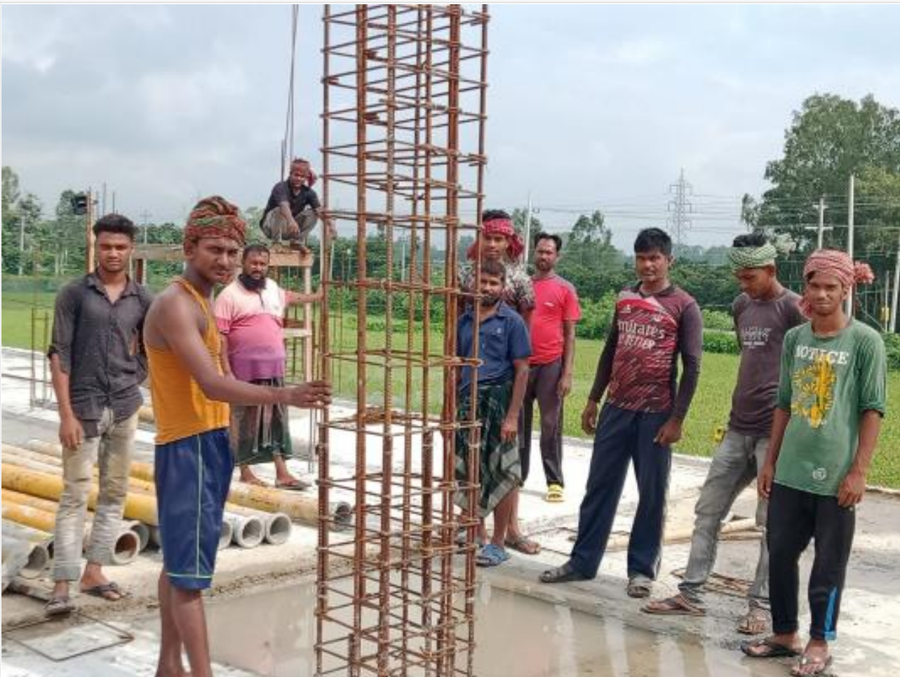
Civil Manpower on 08-07-23
