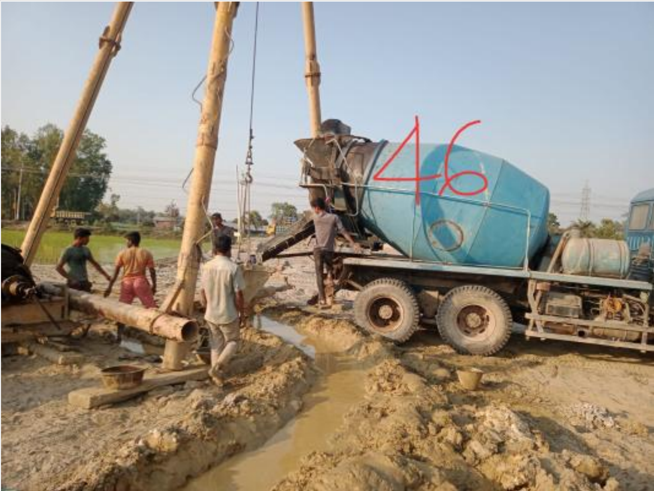
Ready mix concreting of pile on 07-03-23
