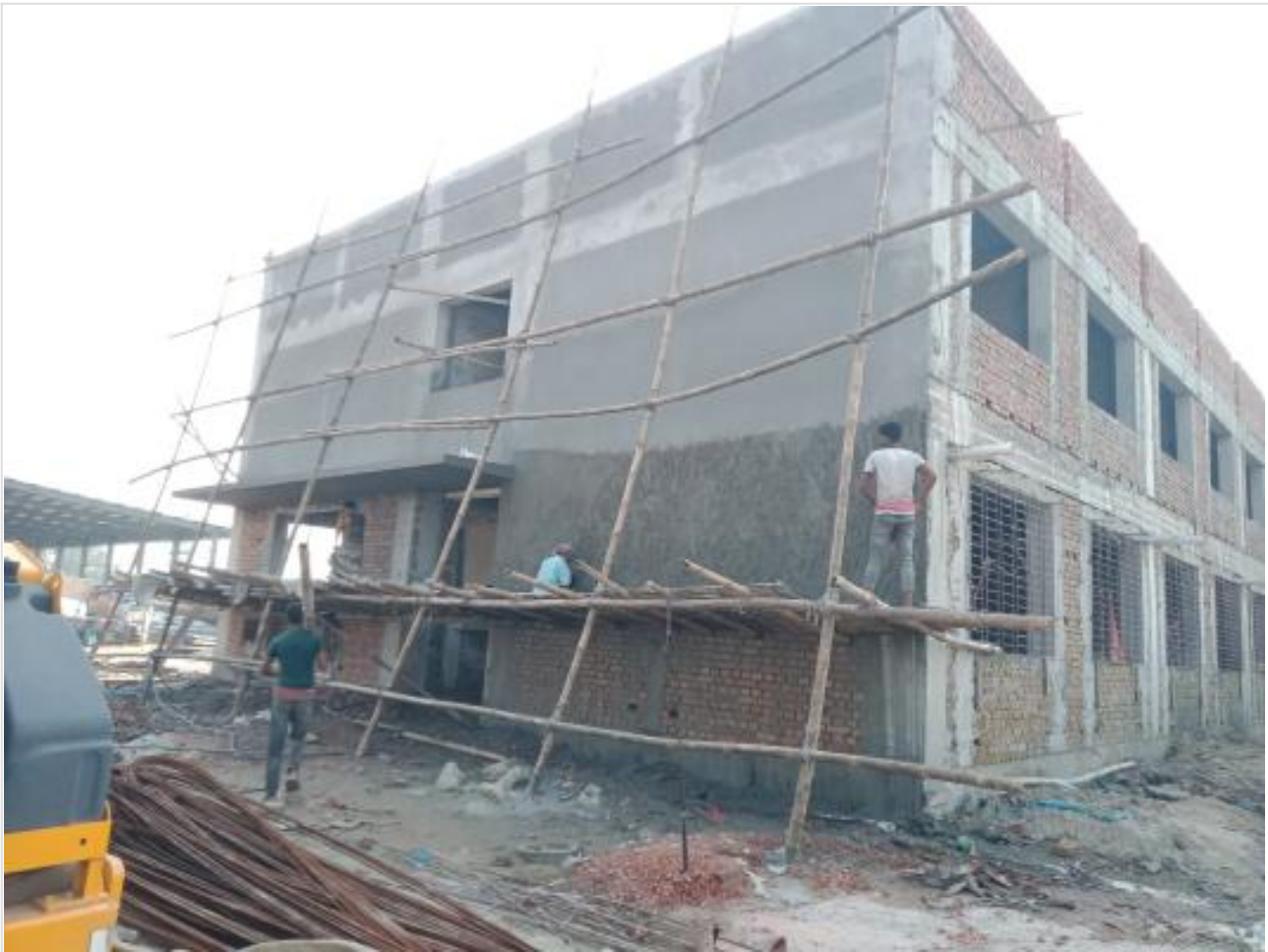
Comp. Bldg. Outside plaster work on 14-10-23
