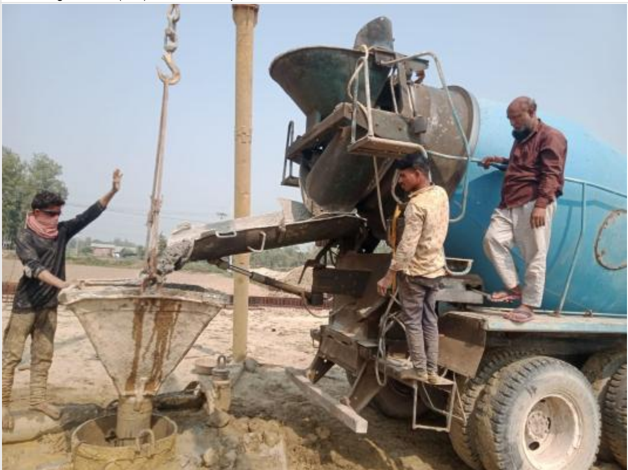
Ready mix concreting of pile on 15-02-23
