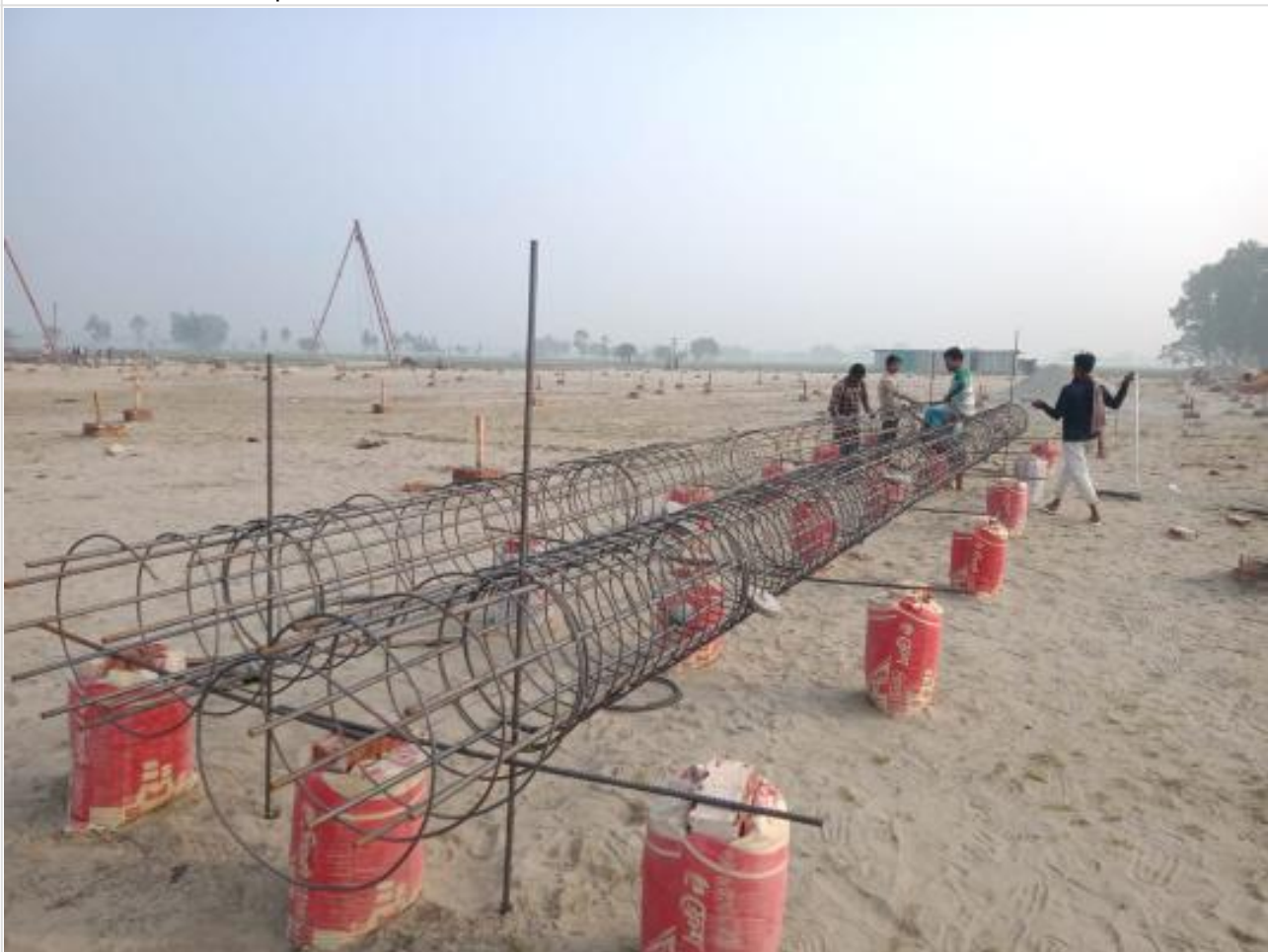
Pile Re-bar Work on 05-02-23
