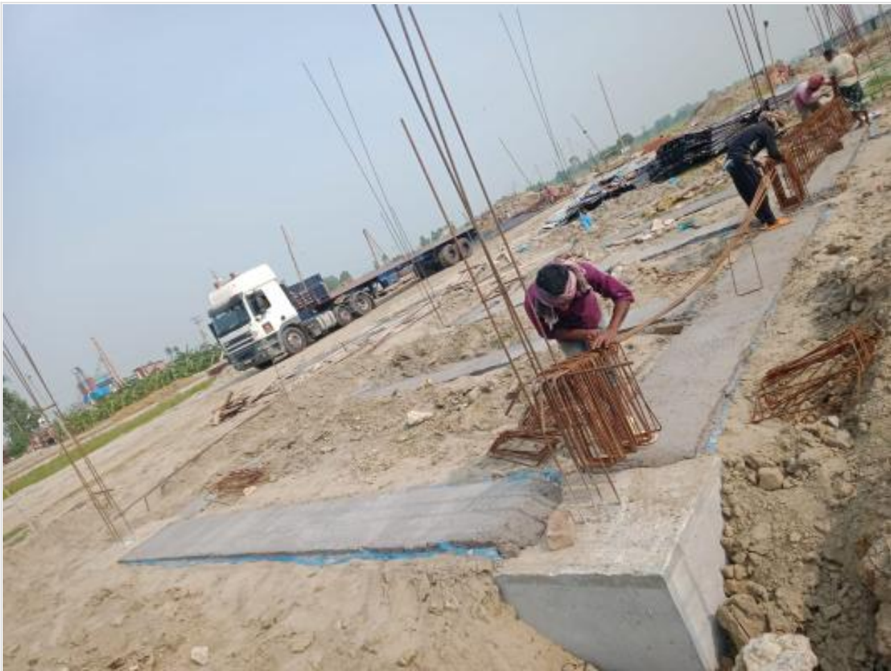
Re-bar work on 13-05-23
