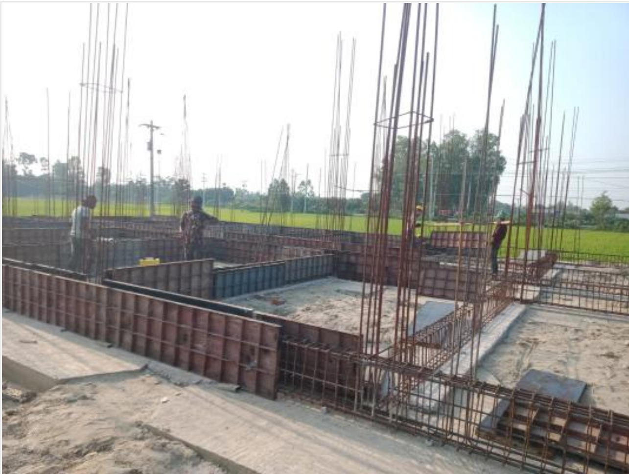
Comp. GB Shuttering on 07-05-23
