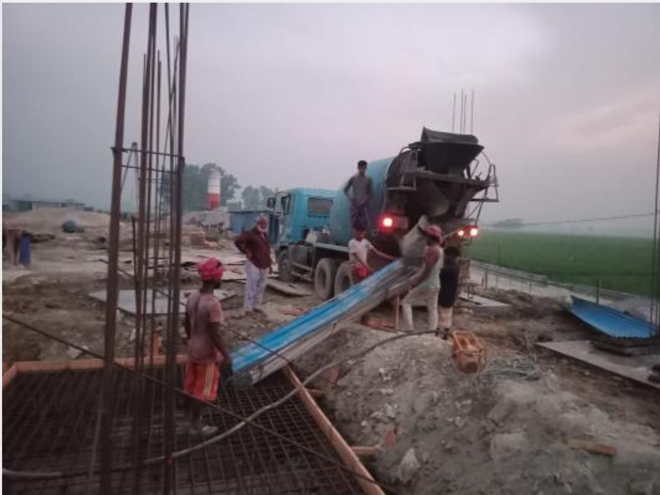
Pile Cap concreting. on 15-04-23
