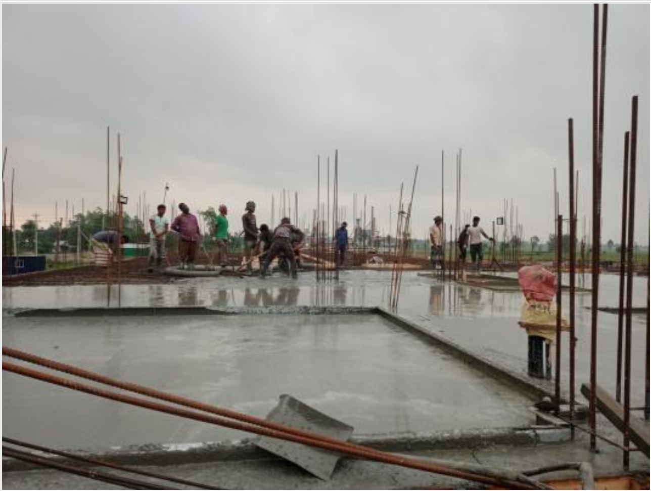
Com. Bldg. 1st floor slab casting on 27-06-23
