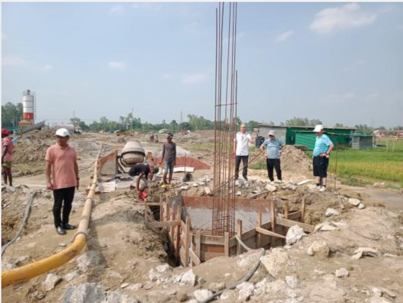
Dorm. Bldg pile cap work on 26-05-23
