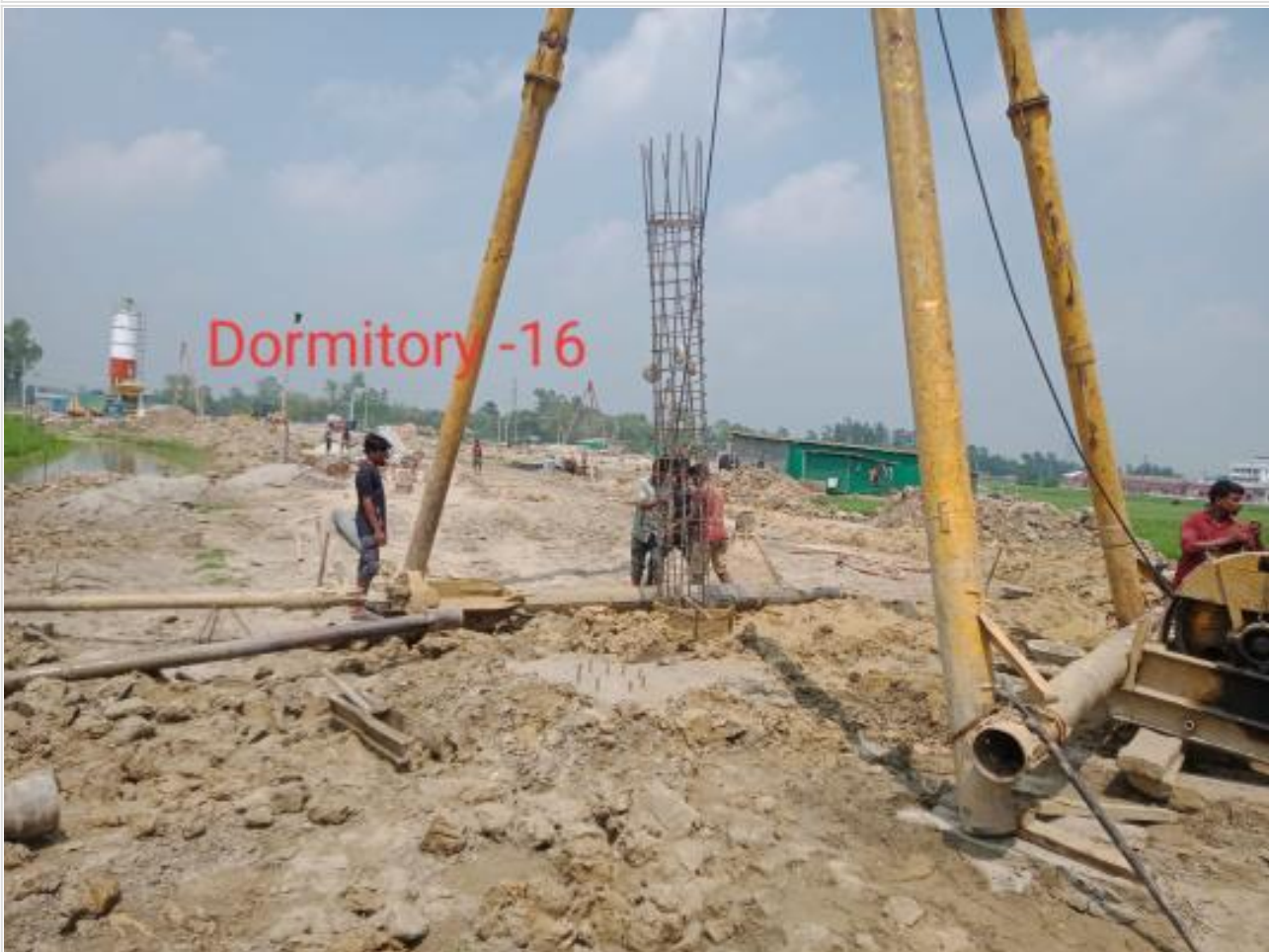
Ready mix concreting of pile on 01-04-23
