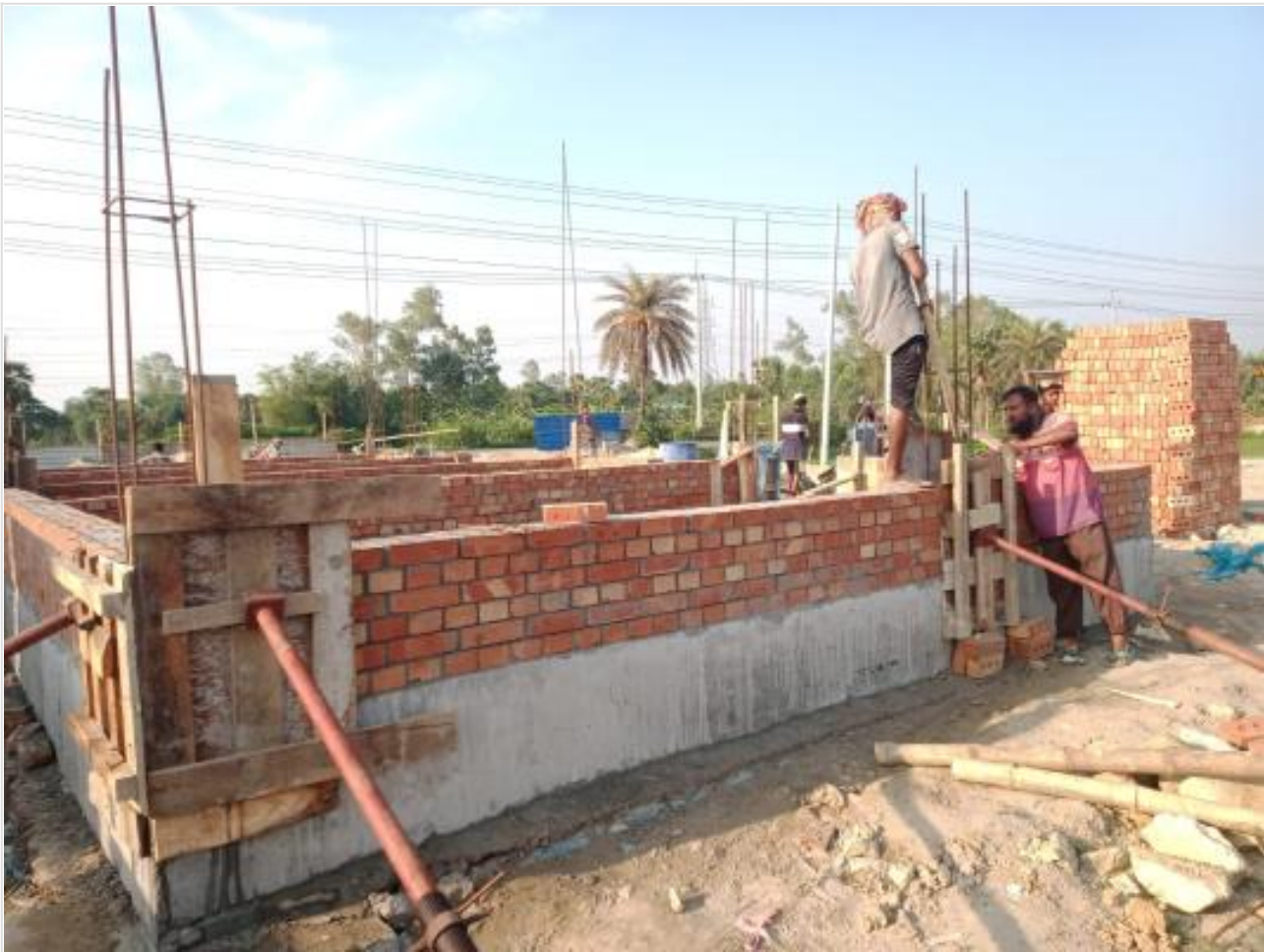
Gate house Brick work on 30-05-23
