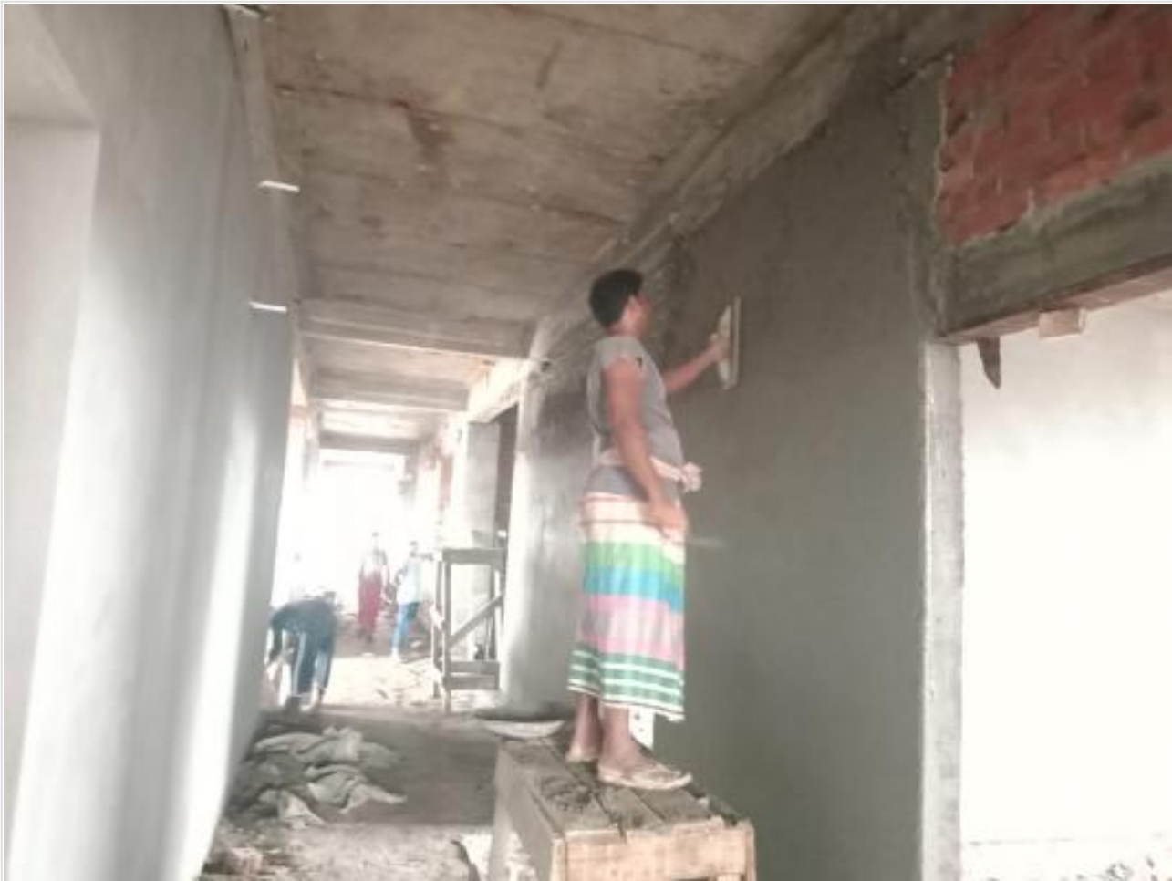
Comp. Bldg plaster work on 26-08-23
