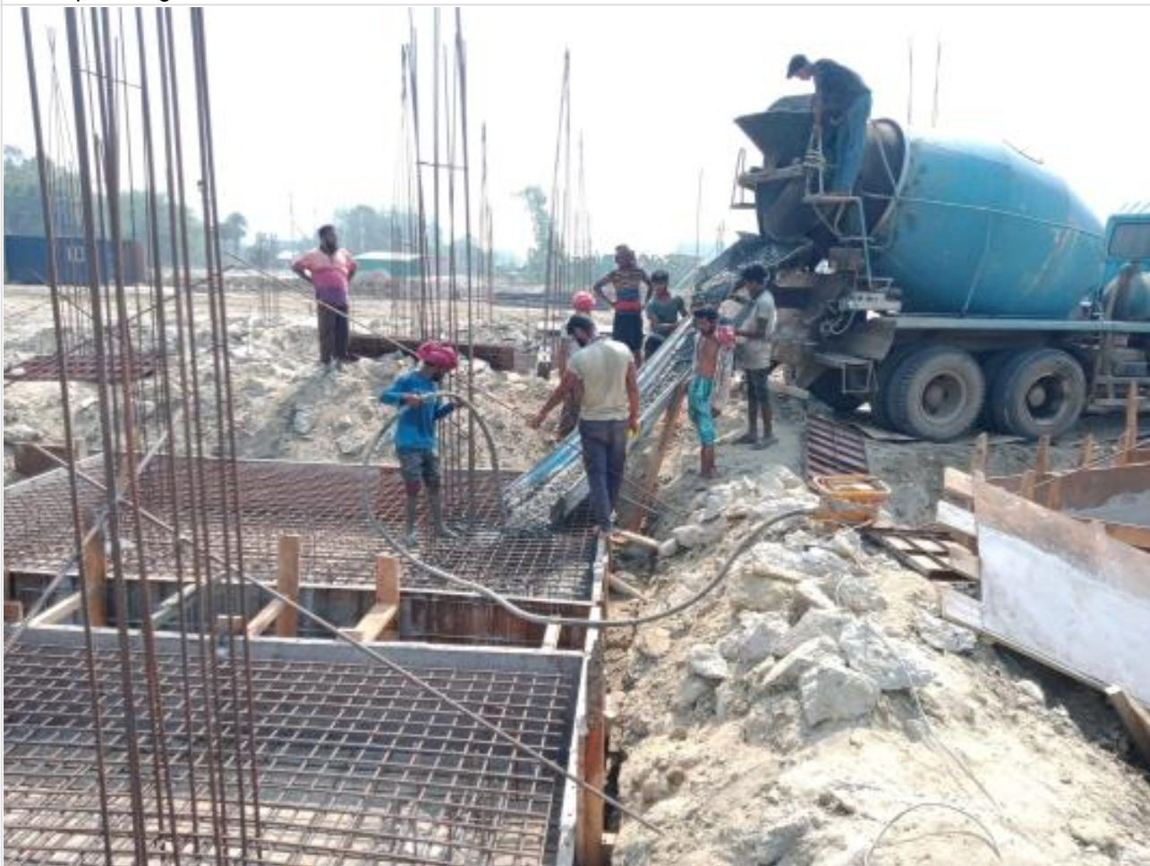
Com. Bldg. Pile cap casting on 17-04-23
