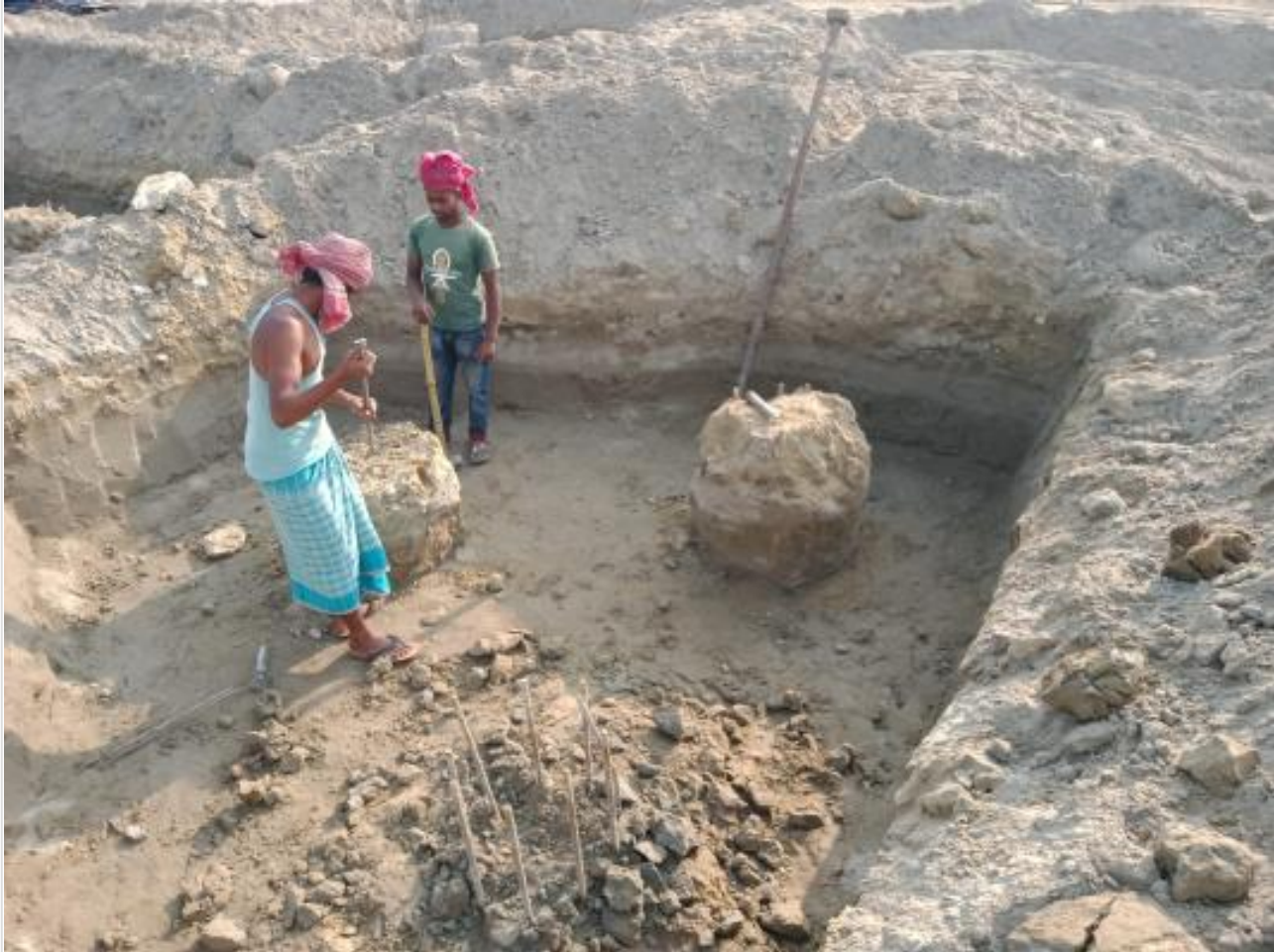
Pile cap earth cutting on 27-03-23
