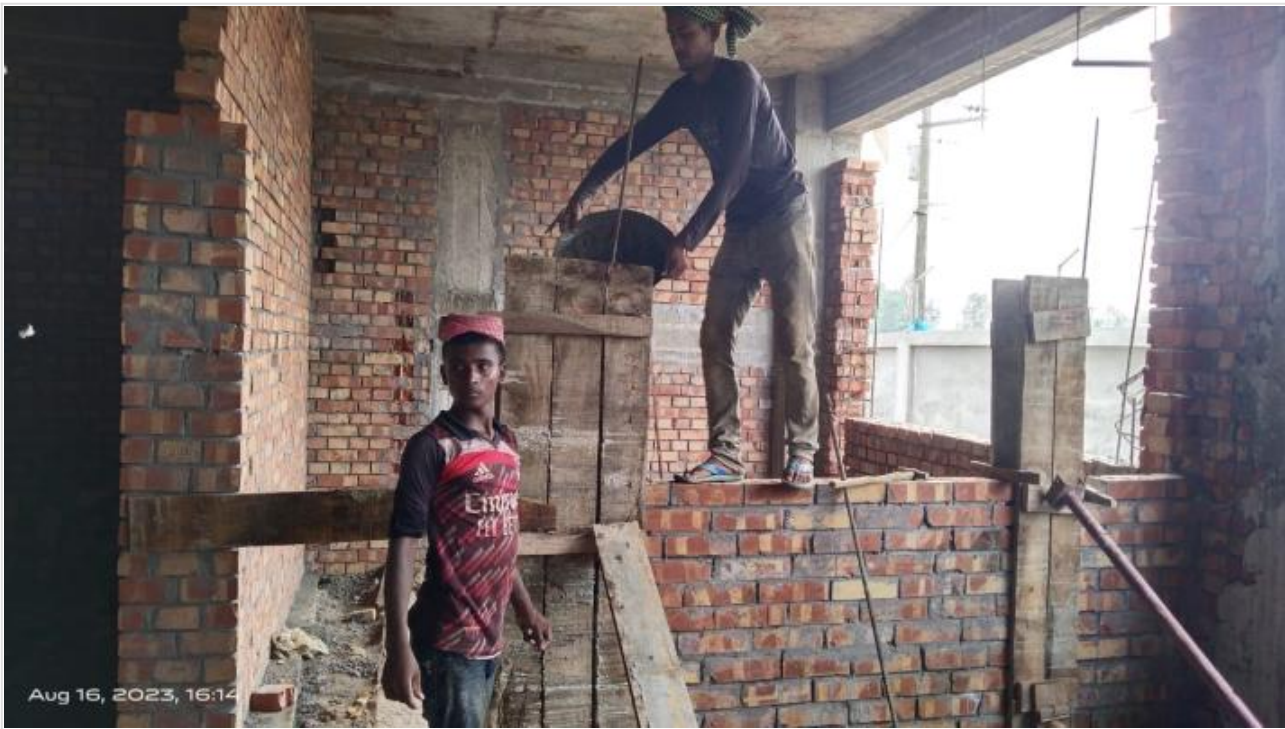
Comp-GF Column Concreting on 16-08-23
