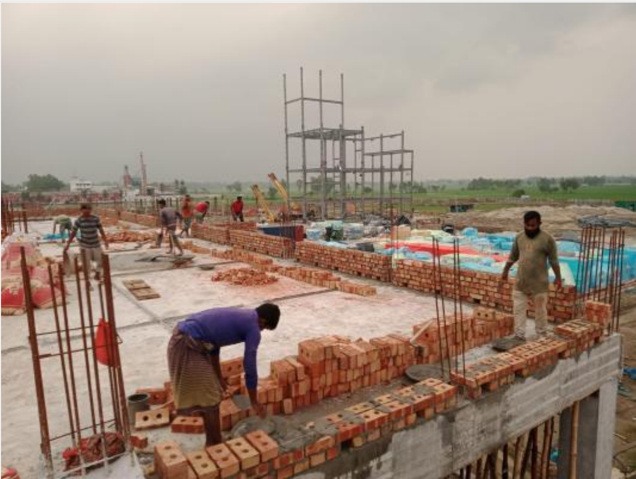
Comp-Parapet Brick-work on 14-08-23
