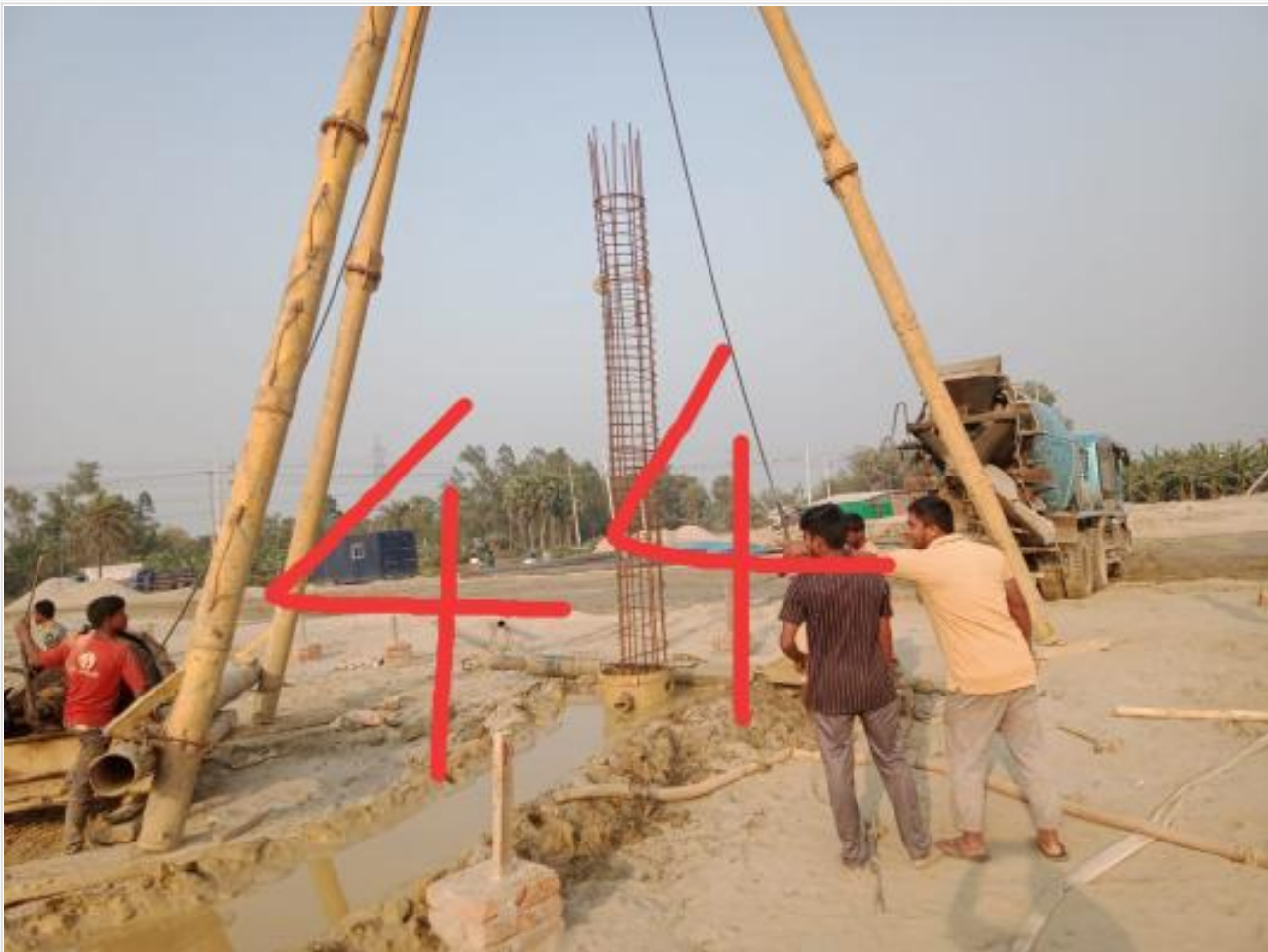
Com. Bldg. 44 pile boring on 05-03-23
