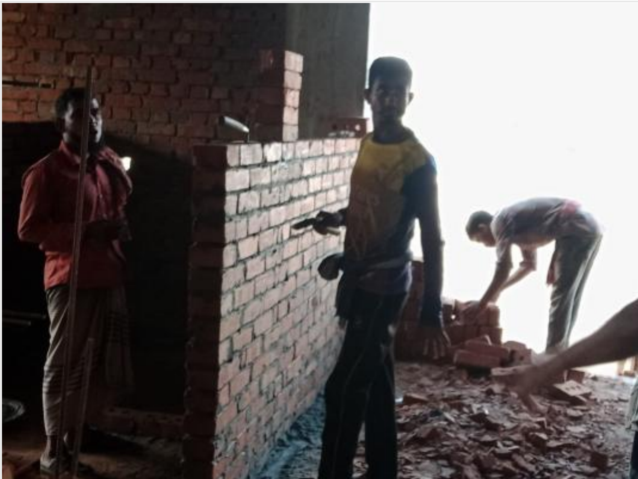
Dorm. Bldg. 1st floor brick work on 13-09-23
