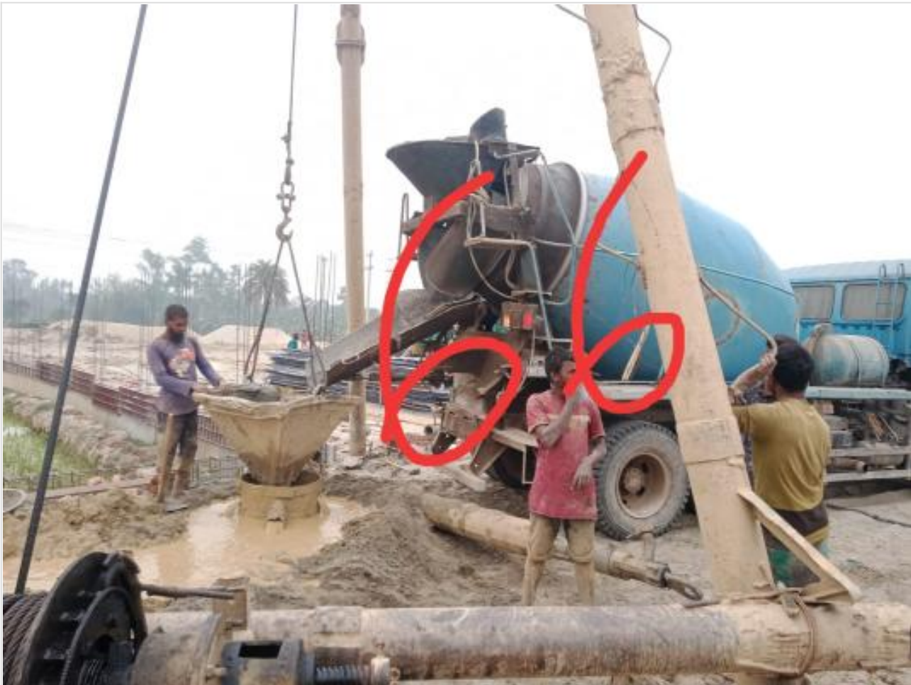
Ready mix concreting of pile on 16-03-23
