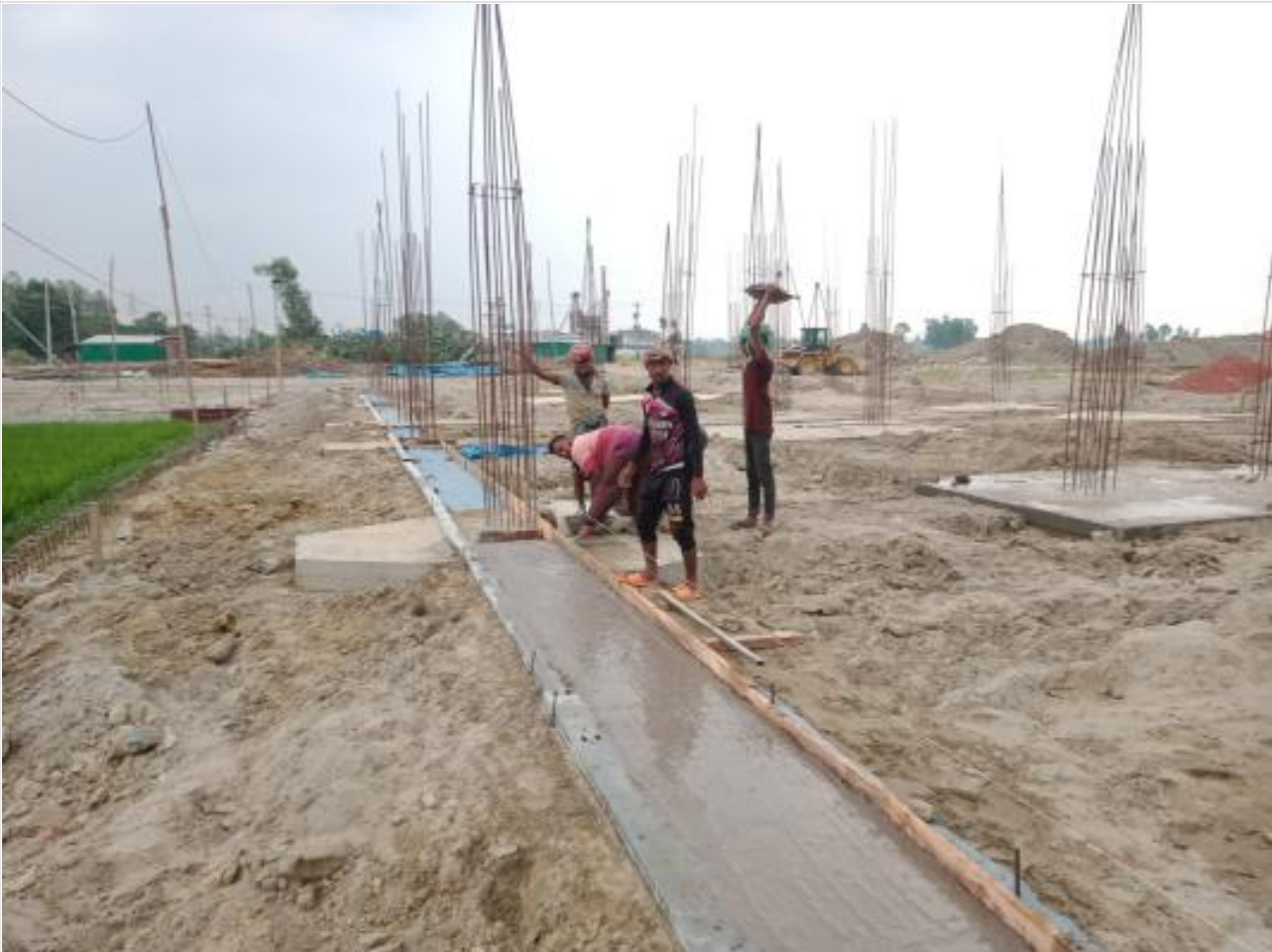
Comp. Bldg. CC casting at GB Bottom on 30-04-23
