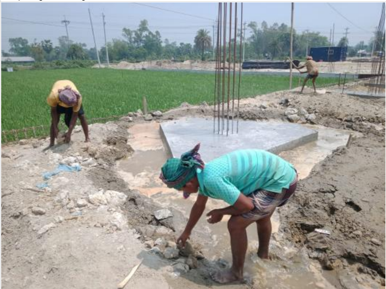
Back filling and levelling dressing. on 19-04-23
