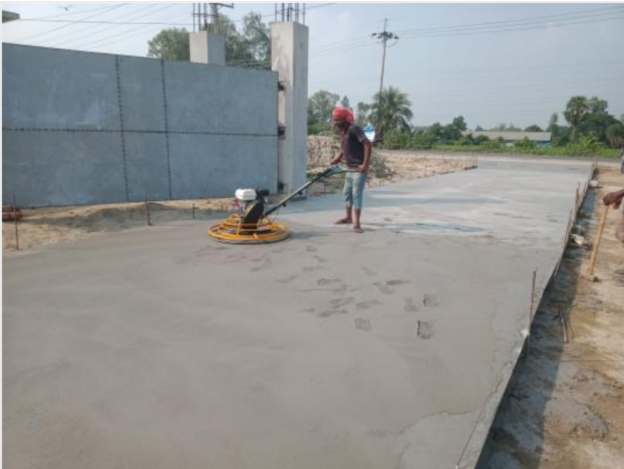
Road casting work on 18-10-23
