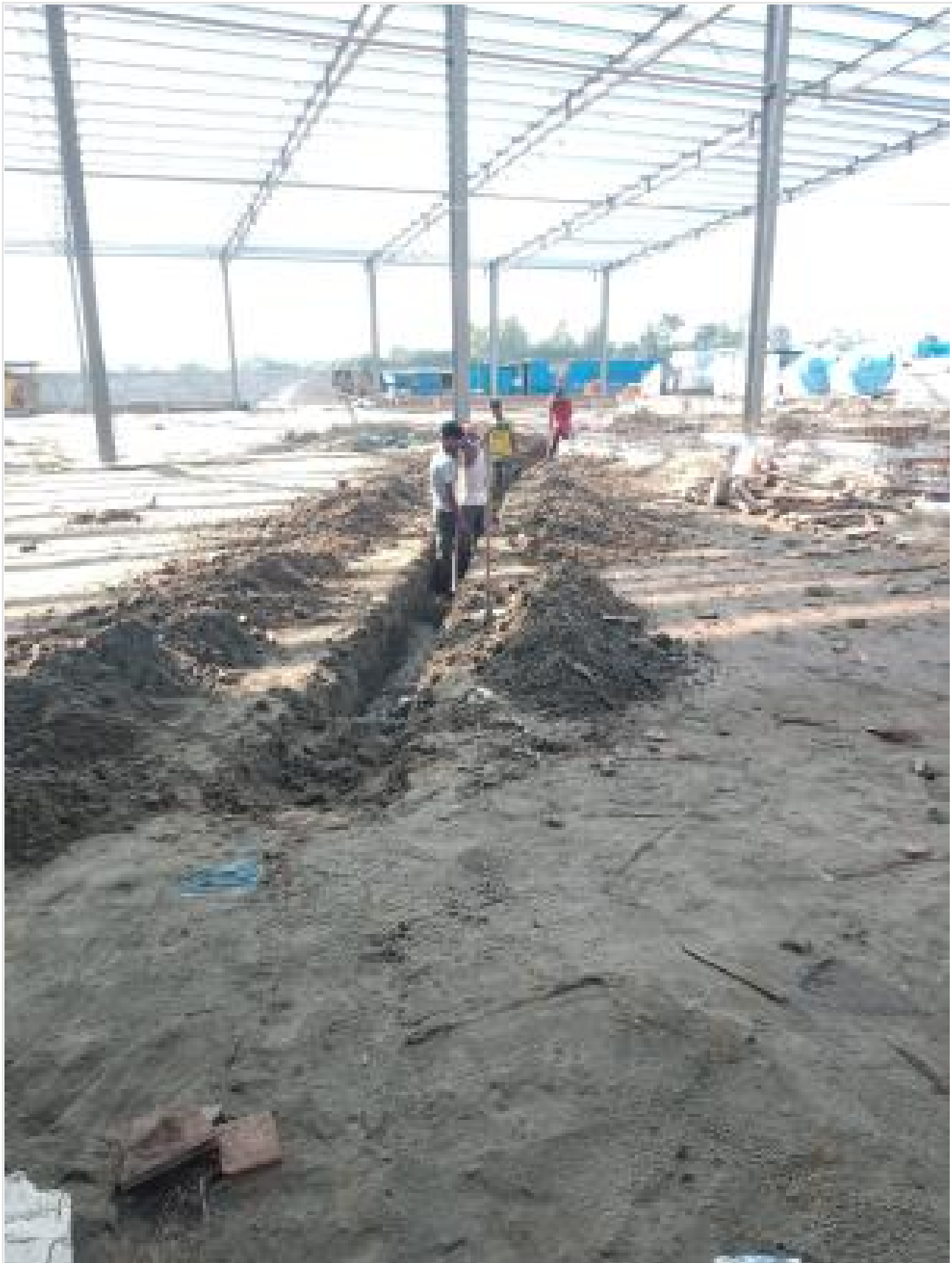
Earth cutting power cable laying on 28-09-23
