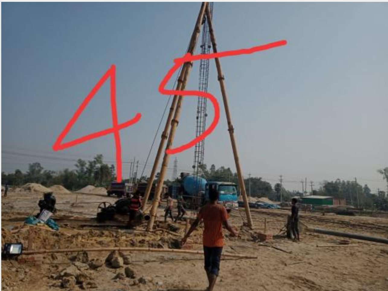
Com. Bldg. 45 Pile Boring on 06-03-23
