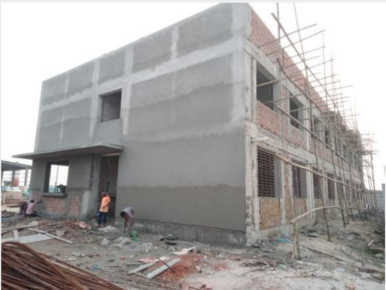
Comp. Bldg. Outside plaster work on 15-10-23
