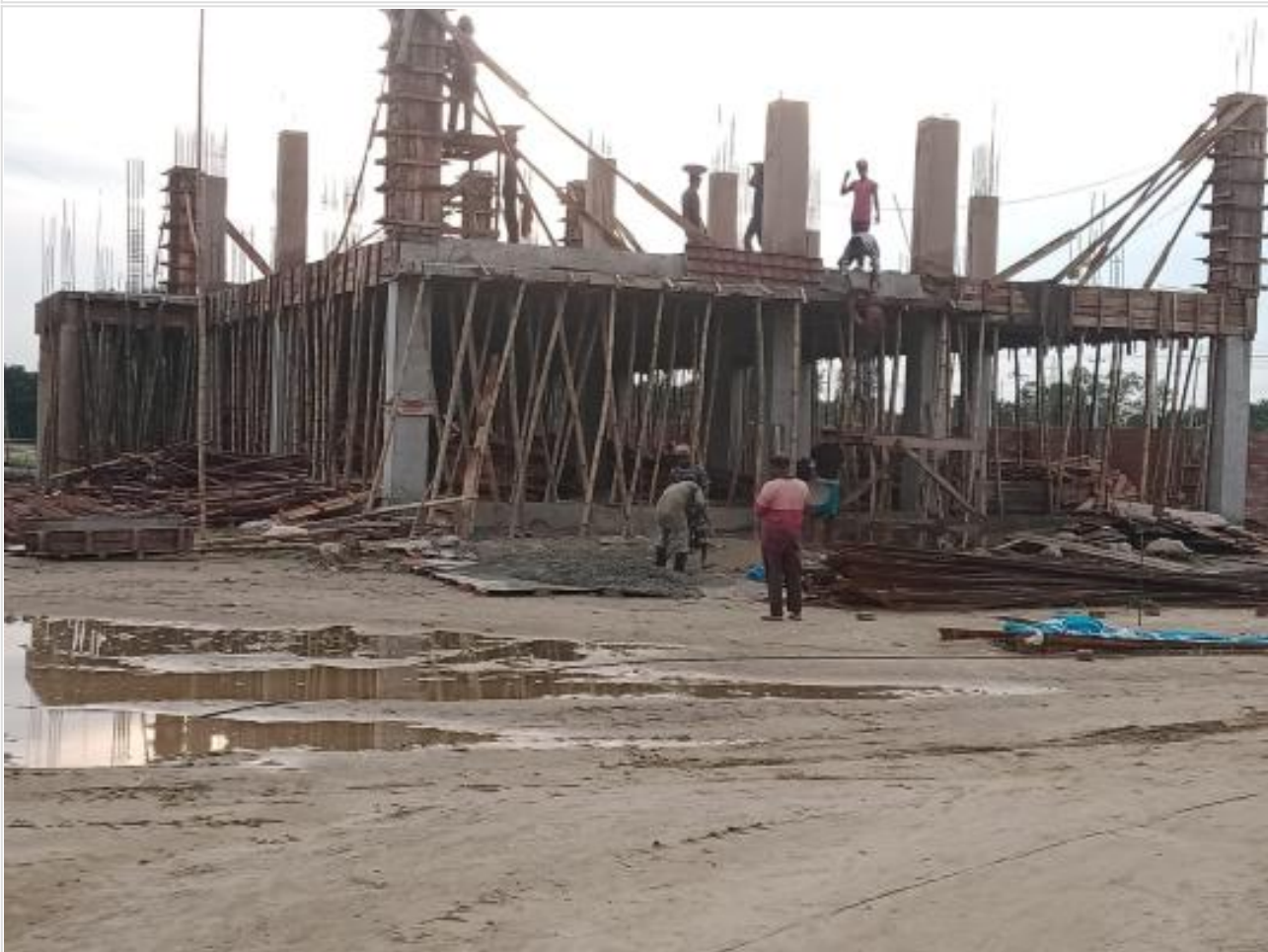
Comp. Bldg. 1st floor column work on 13-07-23
