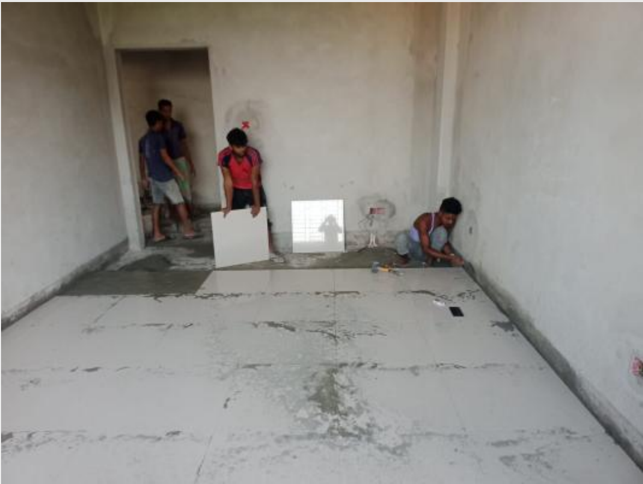
Comp. Bldg. GF Tiles work on 01-11-23
