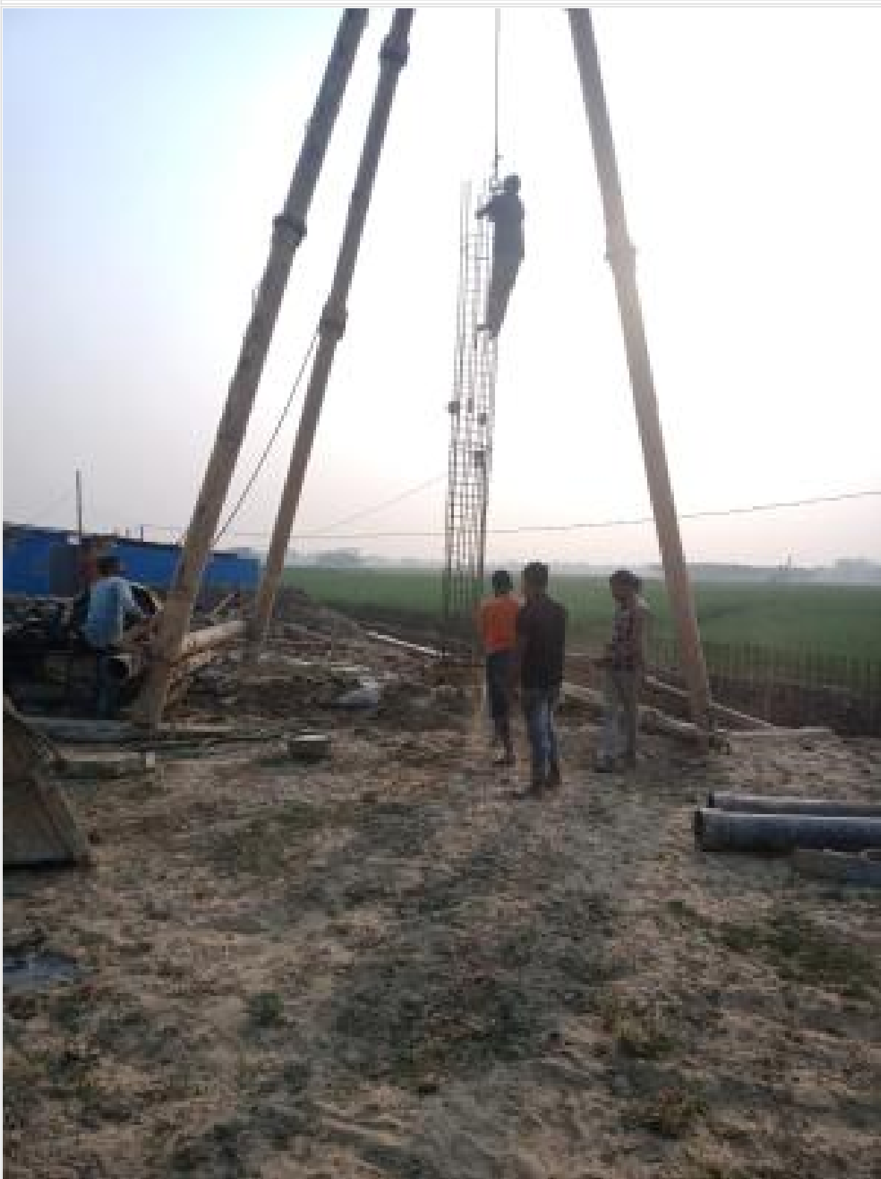
Com. Bldg. 9th pile boring on 16-02-23
