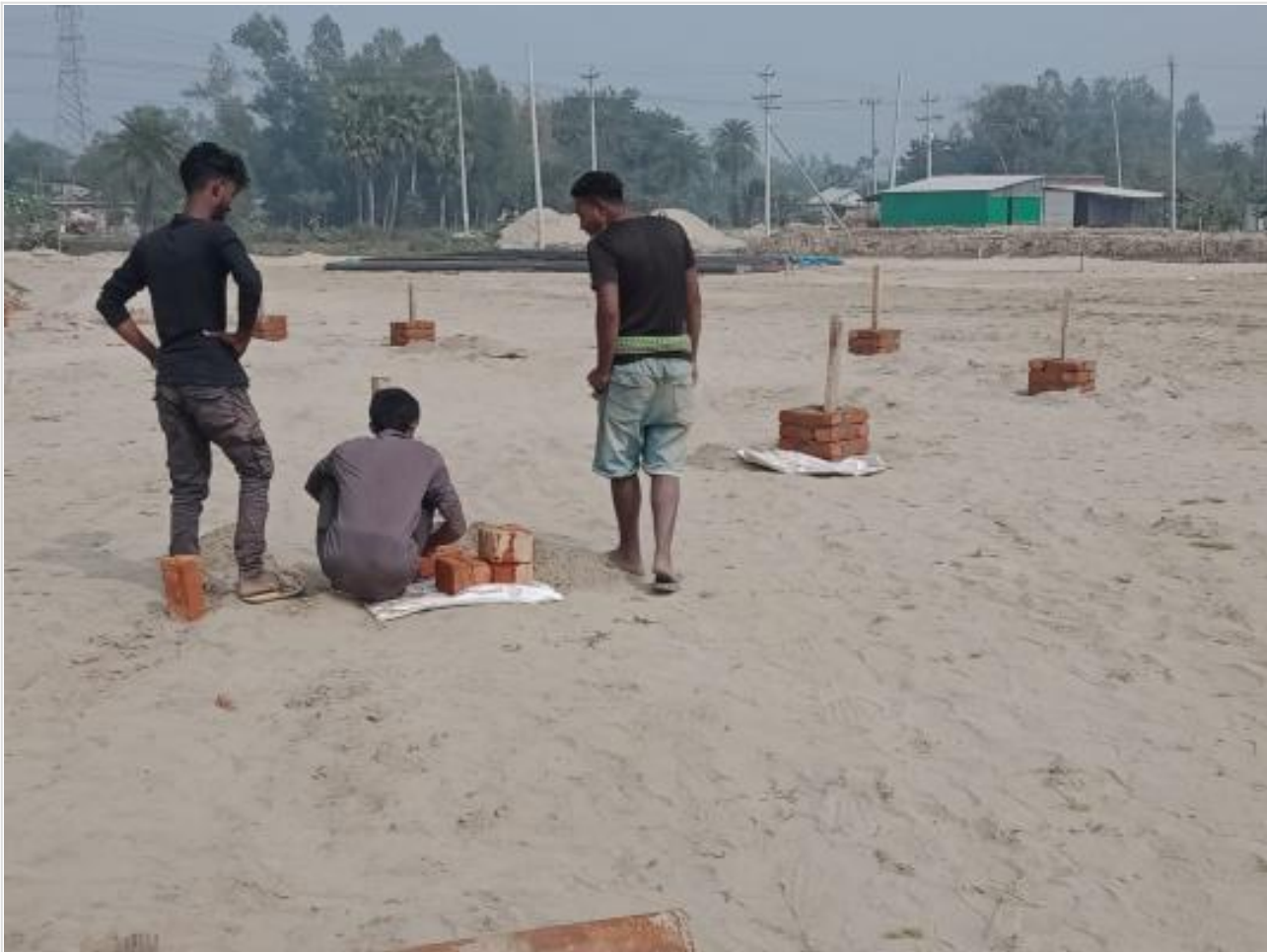
Brick-work around Pile point on 05-02-23
