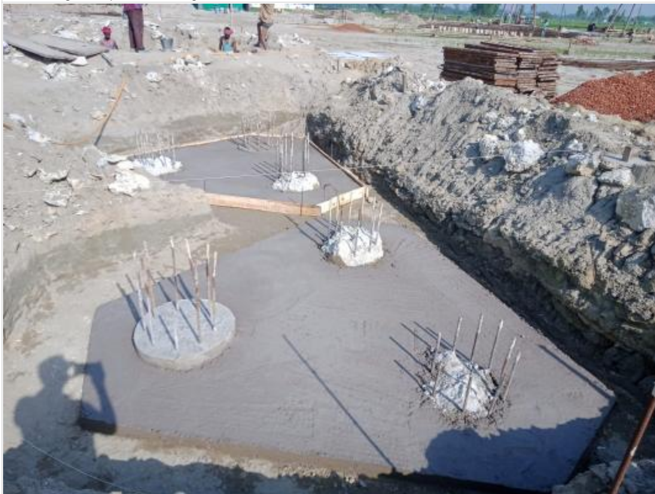
Pile cap CC work on 05-04-23
