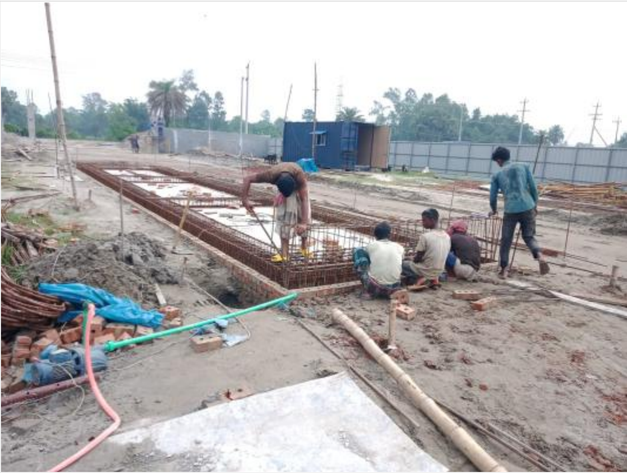
Weighing bridge re-bar work on 11-08-23
