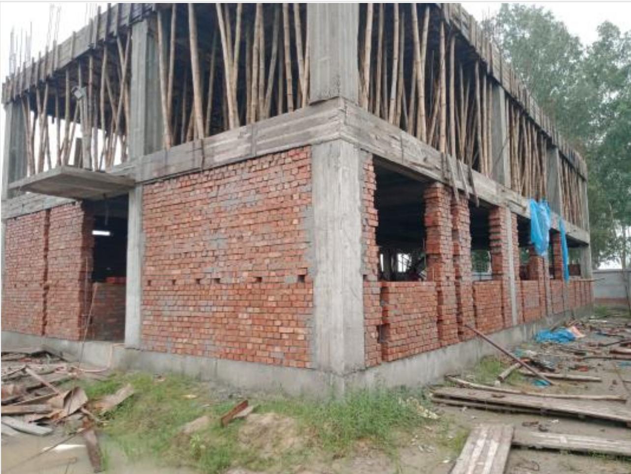
Dorm.Bldg. GF brick work on 25-09-23
