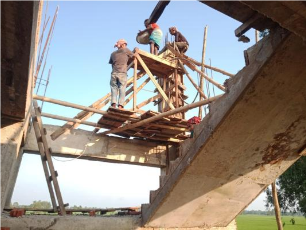
Dorm. Bldg. Roof top column casting on 08-10-23
