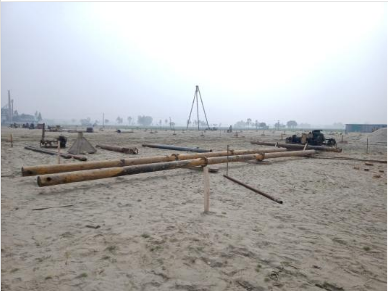
Pile Rig Installing on 31-01-23
