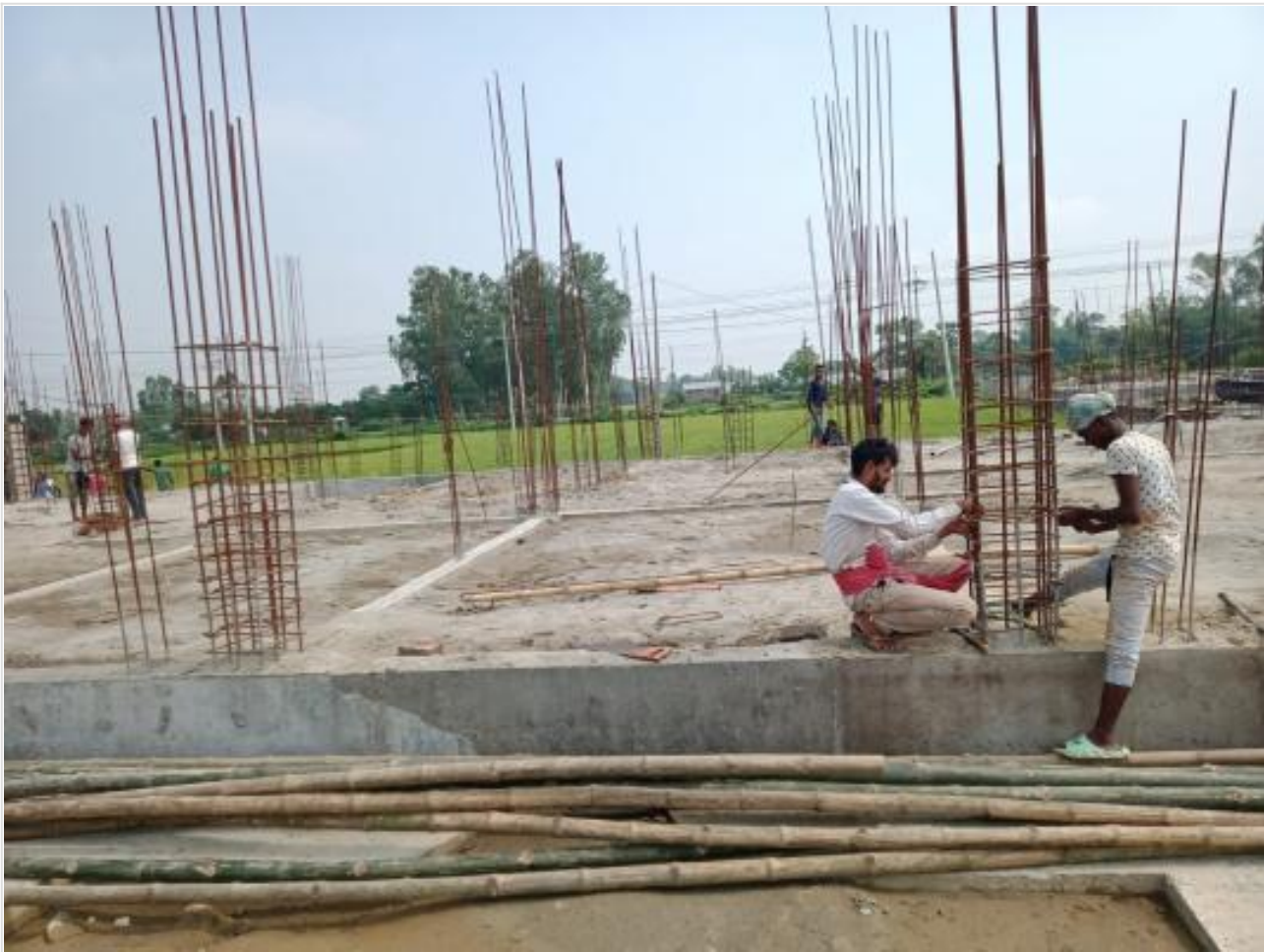
Comp. Bldg column work on 25-05-23
