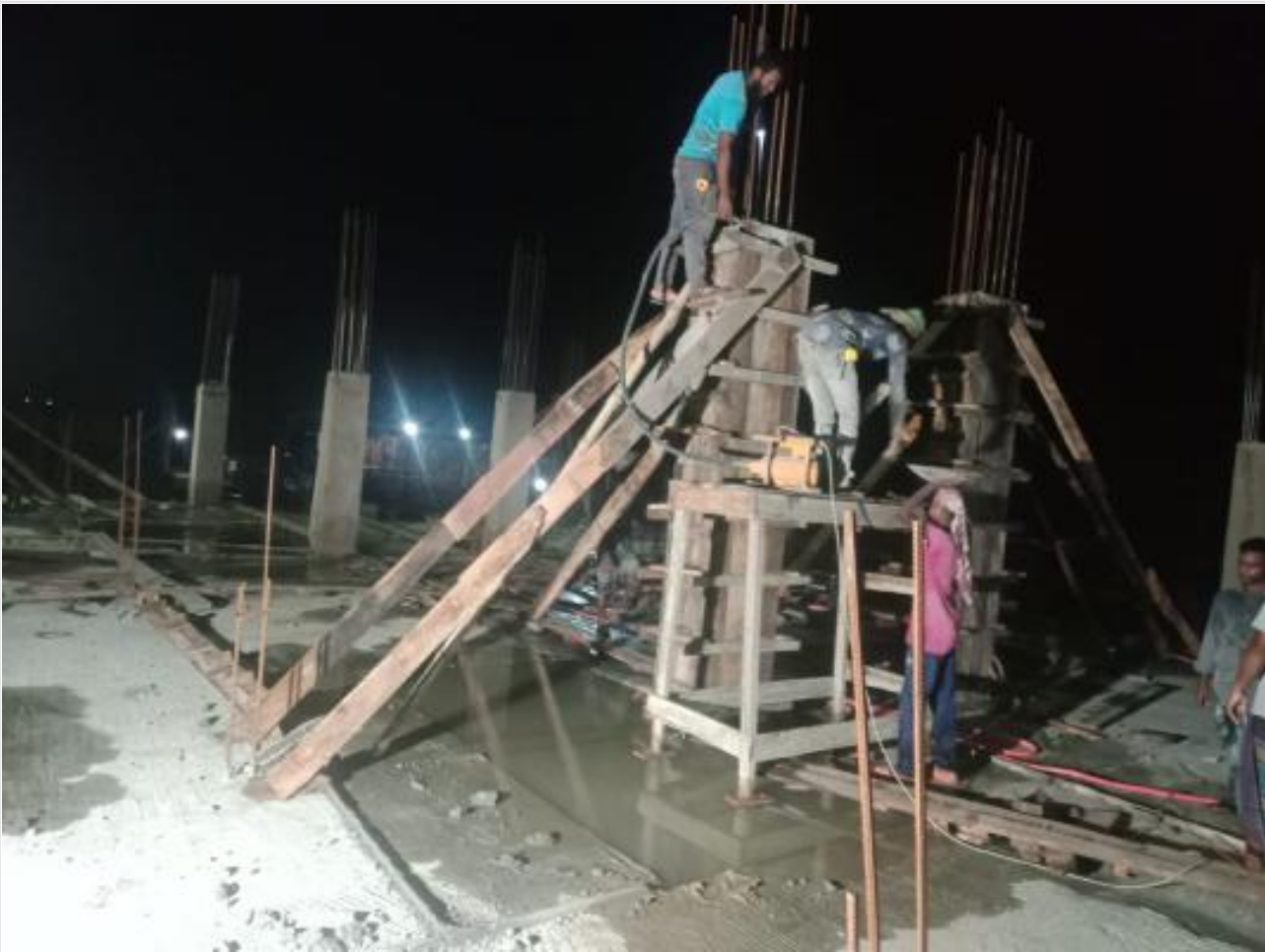
Comp. Bldg 1st floor column casting on 13-07-23
