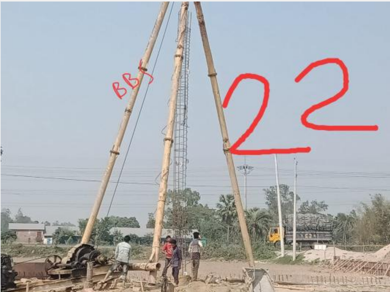
Ready mix concreting of pilewort on 22-02-23
