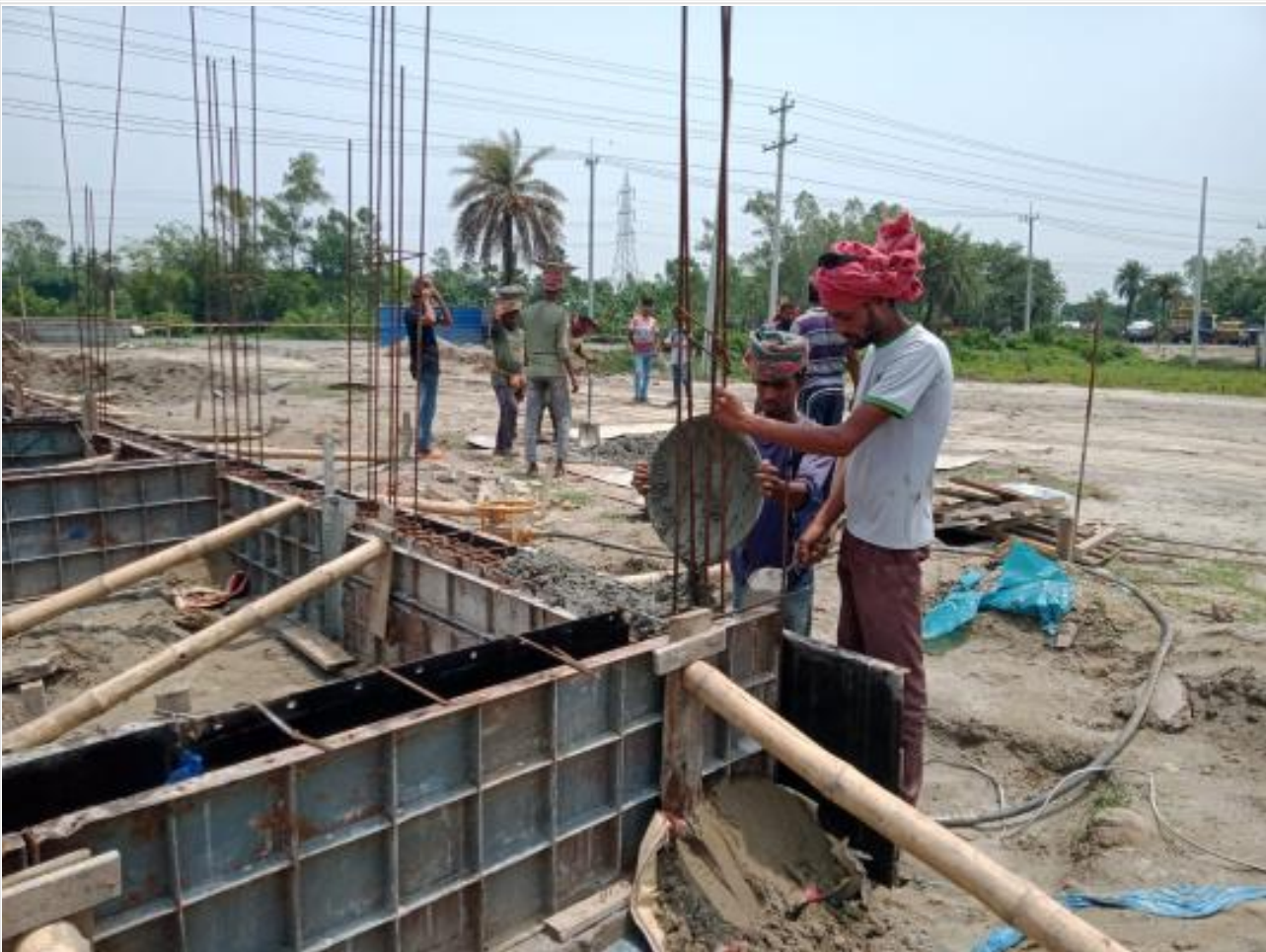
Guard House GB Casting on 18-05-23
