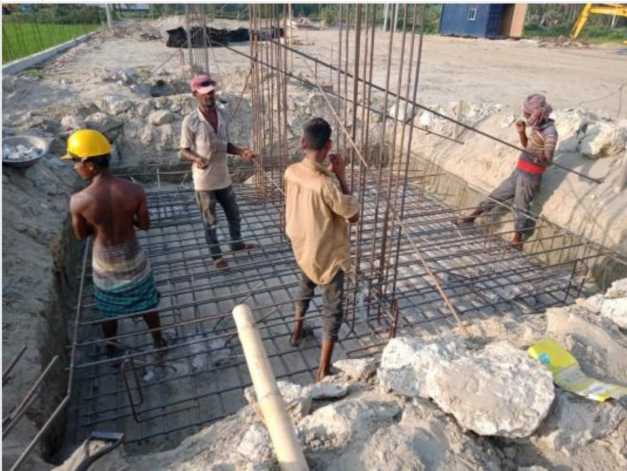
Pile cap rebar work on 14-04-23
