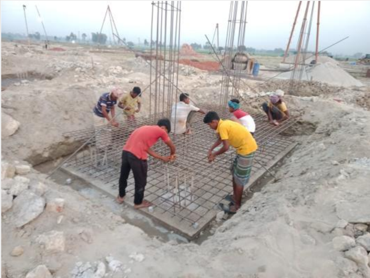
Com. Bldg. Pile cap work on 10-04-23
