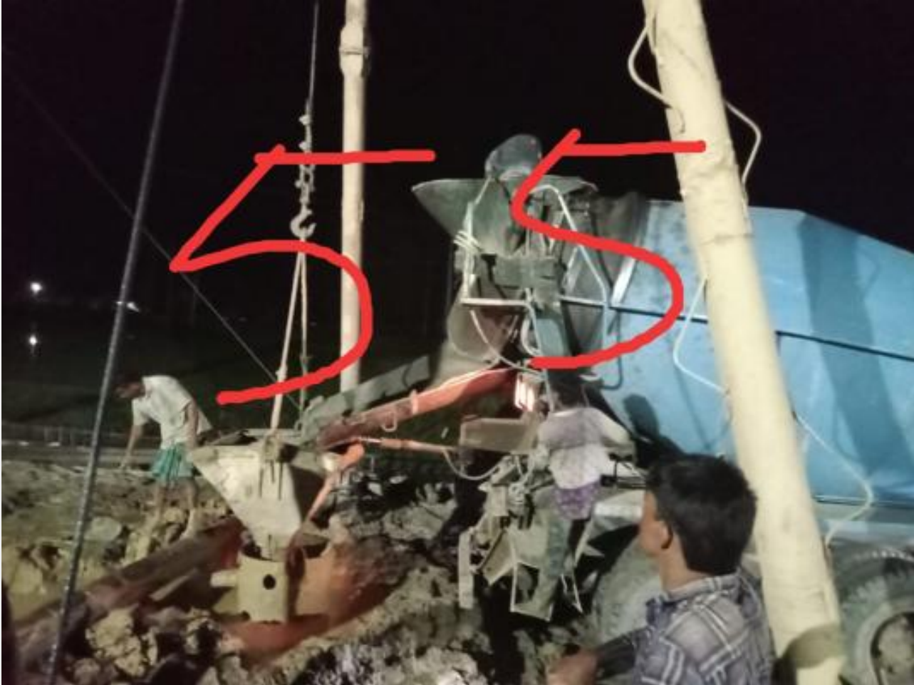
Ready mix concreting of pile on 11-03-23
