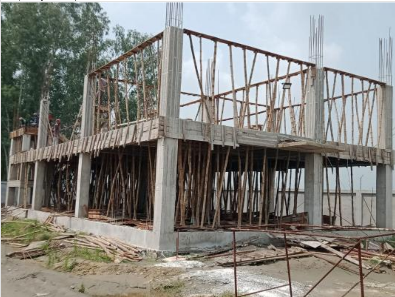
Dorm. Bldg. 2nd floor shuttering on 29-08-23
