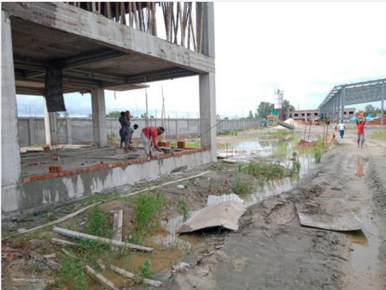
Dormitory GF-Brick Work on 20-09-23
