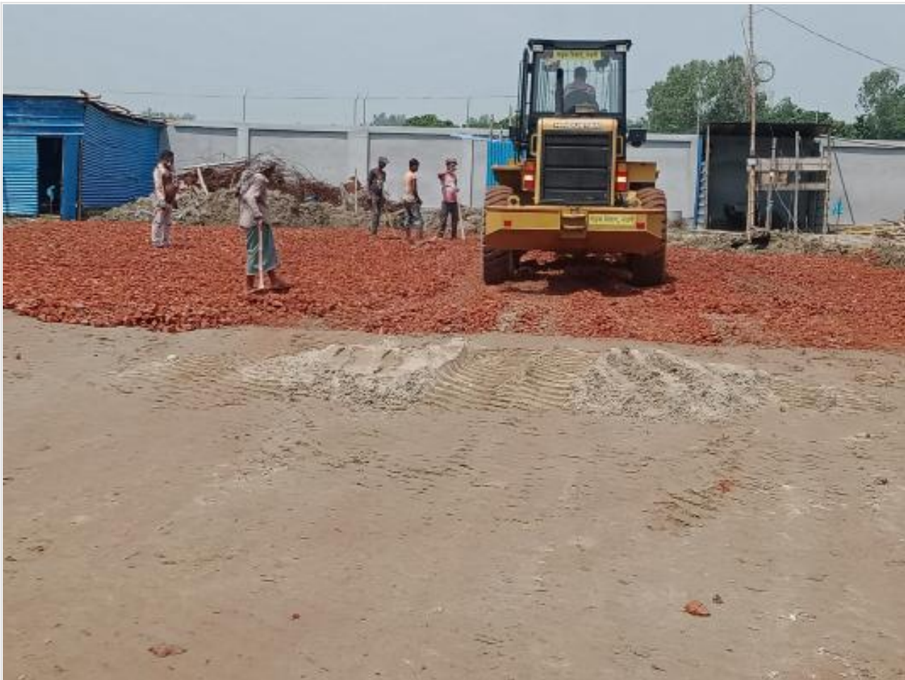
Road Sub-base work on 30-08-23
