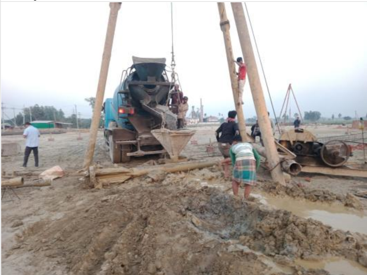
Ready mix concreting of pile on 14-02-23
