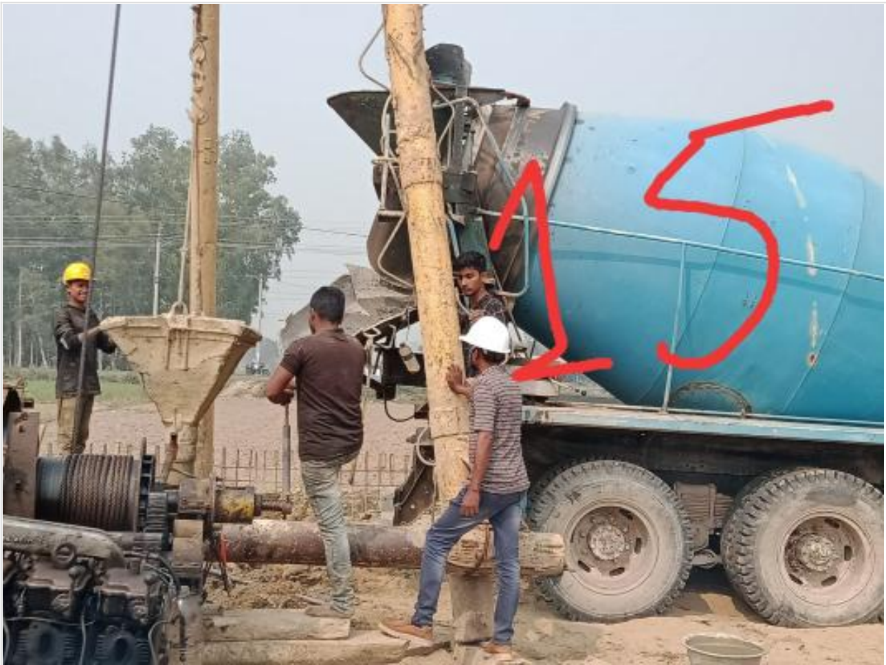
Ready mix concreting of pile on 19-02-23
