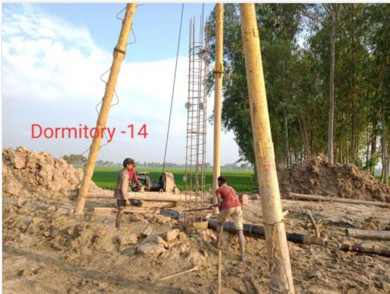
Ready mix concreting of pile on 31-03-23
