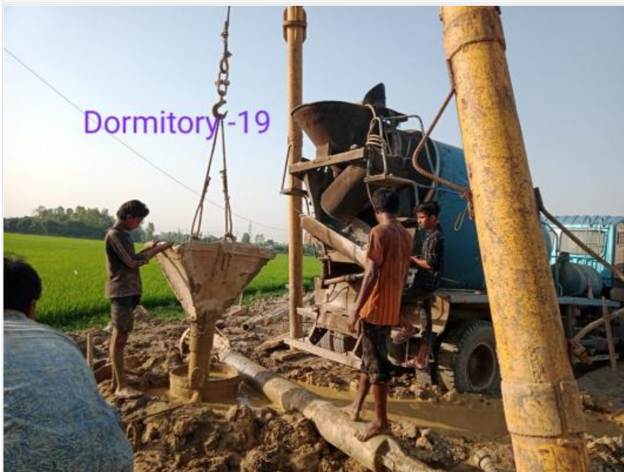
Pile cap bottom cc casting. on 04-04-23
