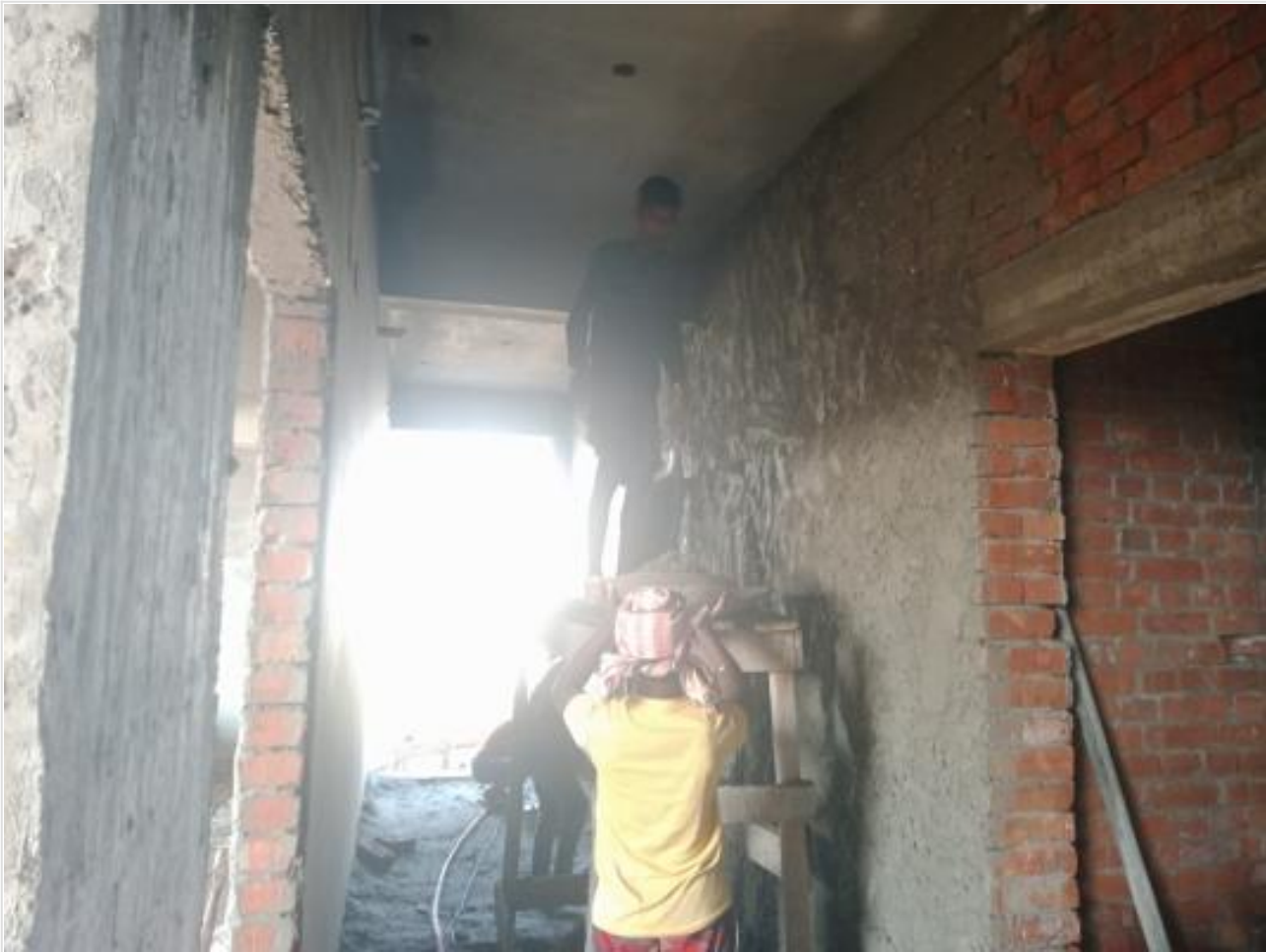
Dorm. Bldg. Plaster work on 02-11-23
