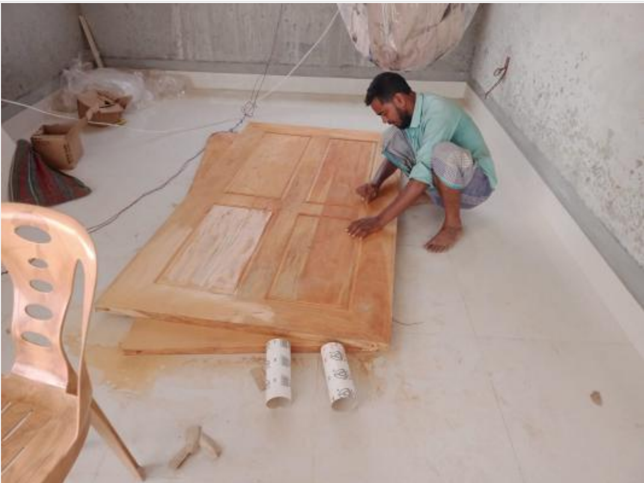
Comp. Bldg. Door shutter work on 26-10-23
