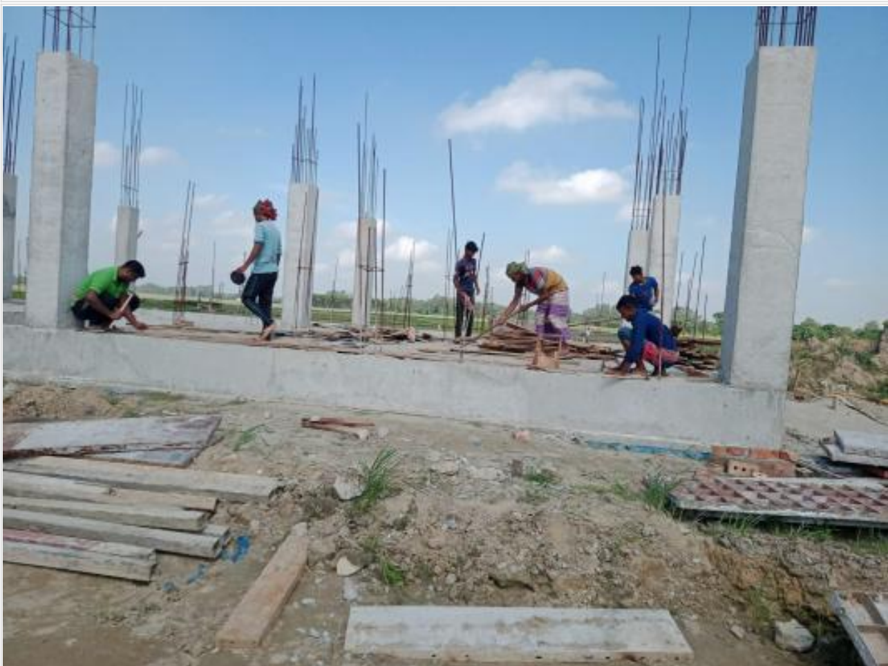
Dorm. Bldg. Floor levelling work on 20-07-23
