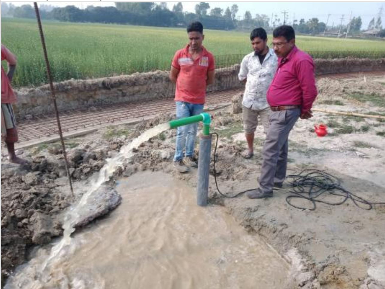
Deep tube well sinking on 01-02-23
