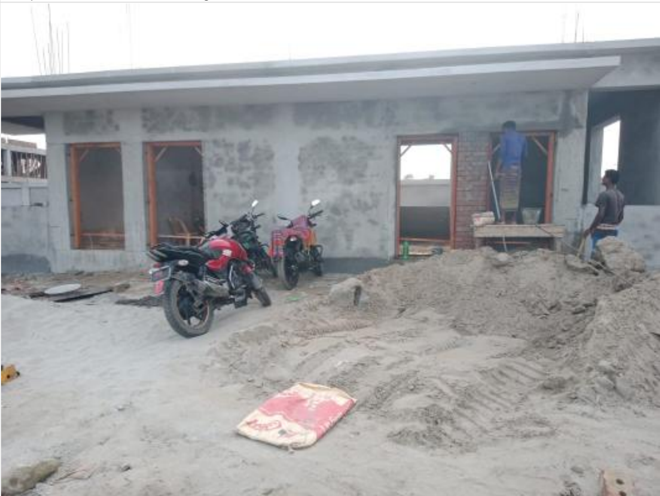
Gate House-Door Frame Fixing on 20-08-23
