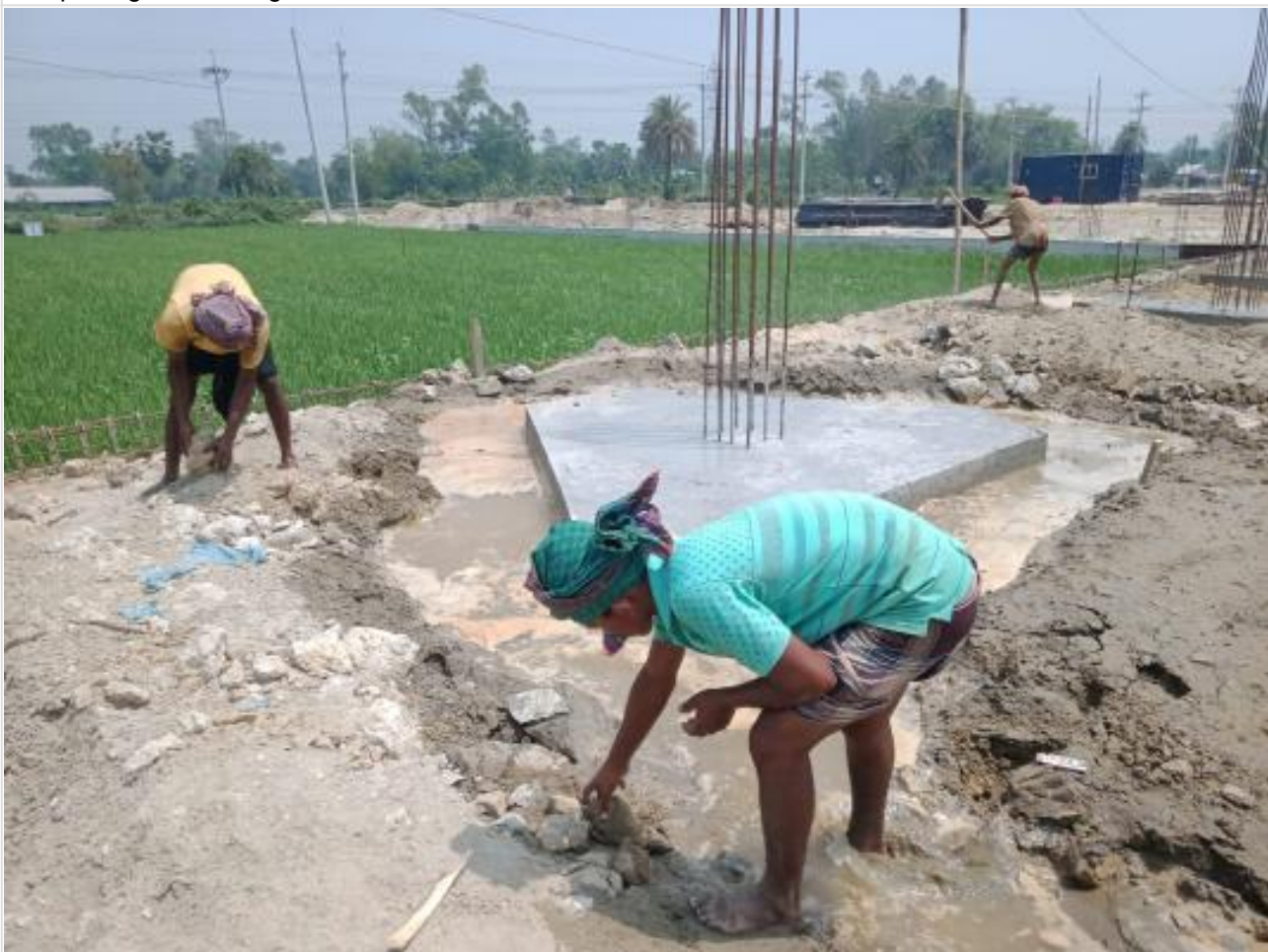
Back filling and levelling dressing. on 19-04-23
