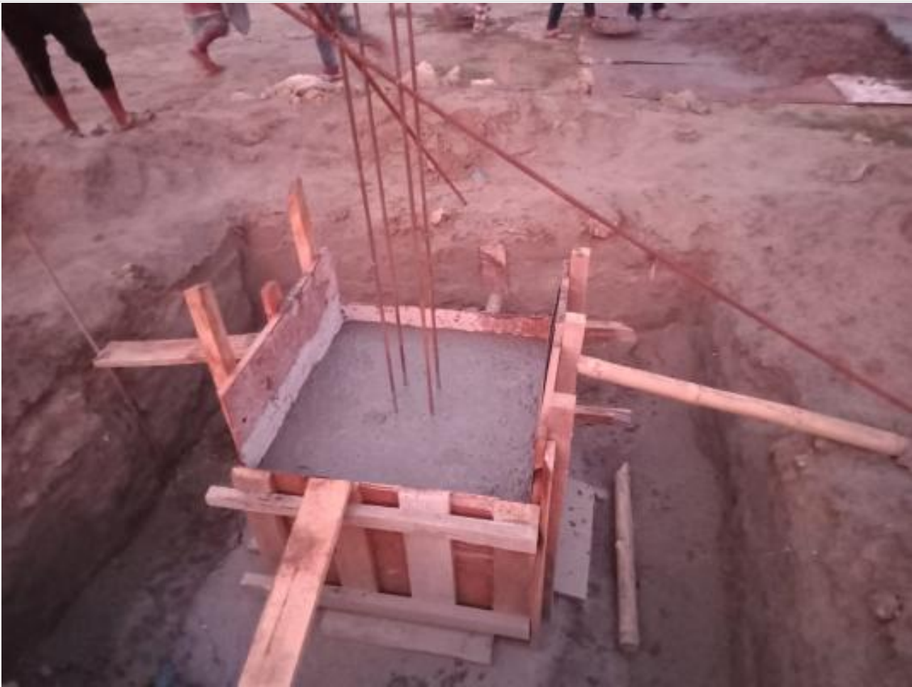
Gate house pile cap casting on 12-05-23
