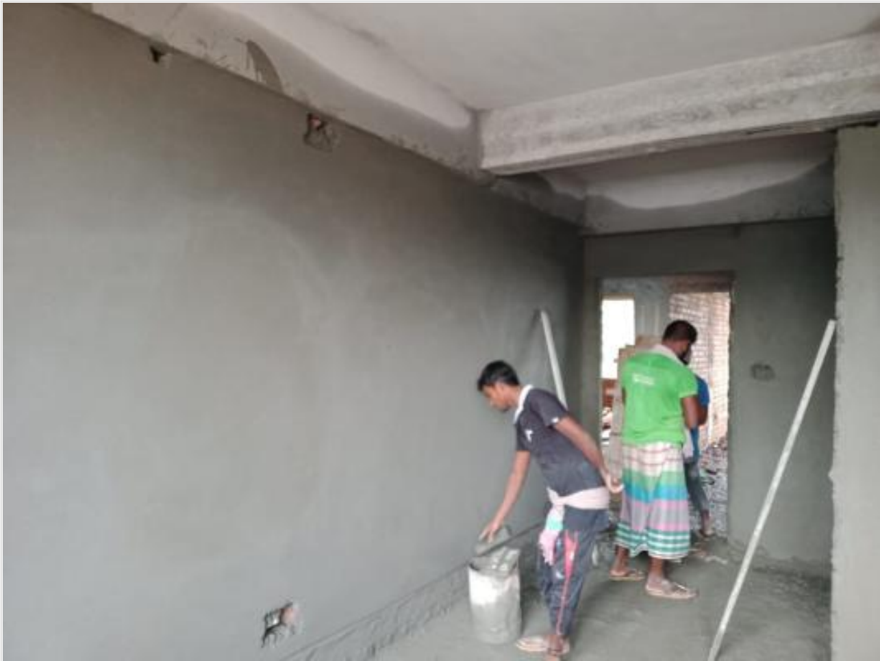
Comp. Bldg 1st fplaster work on 21-09-23
