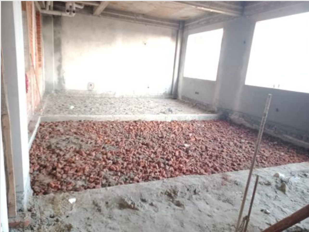
Comp. GF Cushion concreting on 15-09-23
