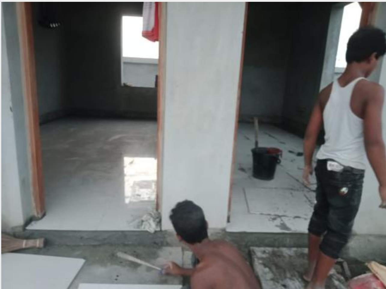
Gats house tiles work on 26-09-23
