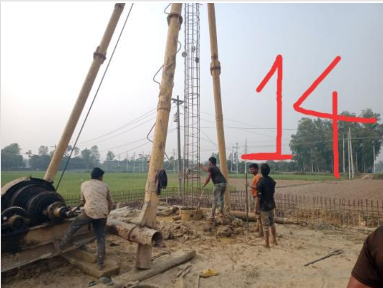
Com. Bldg. 14th pile boring on 18-02-23
