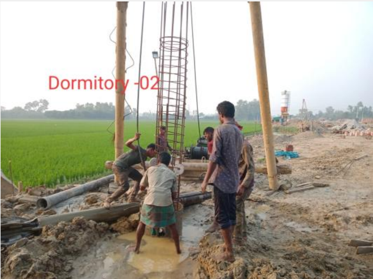
Pile head breaking on 24-03-23
