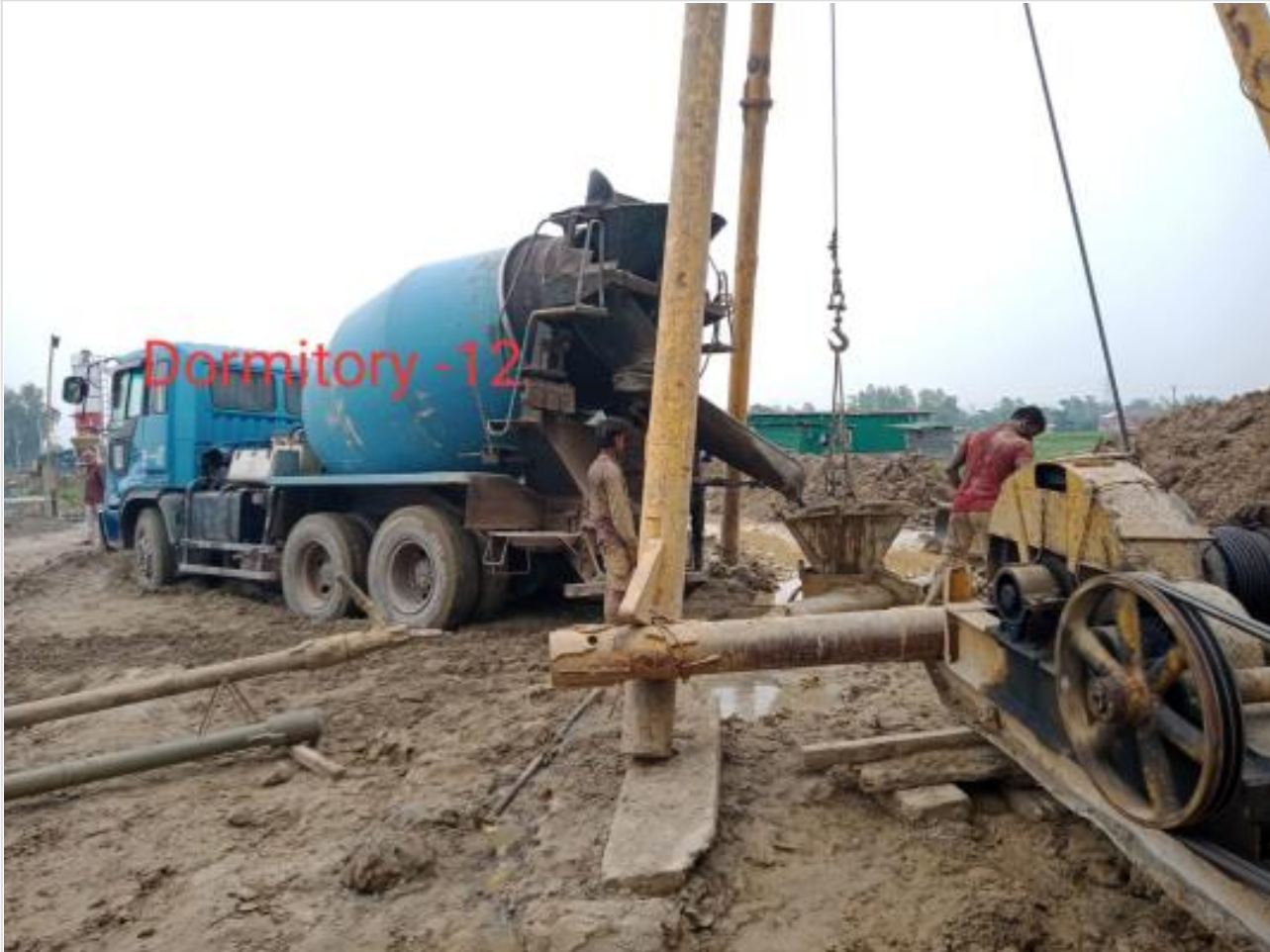
Ready mix concreting of pile on 31-03-23
