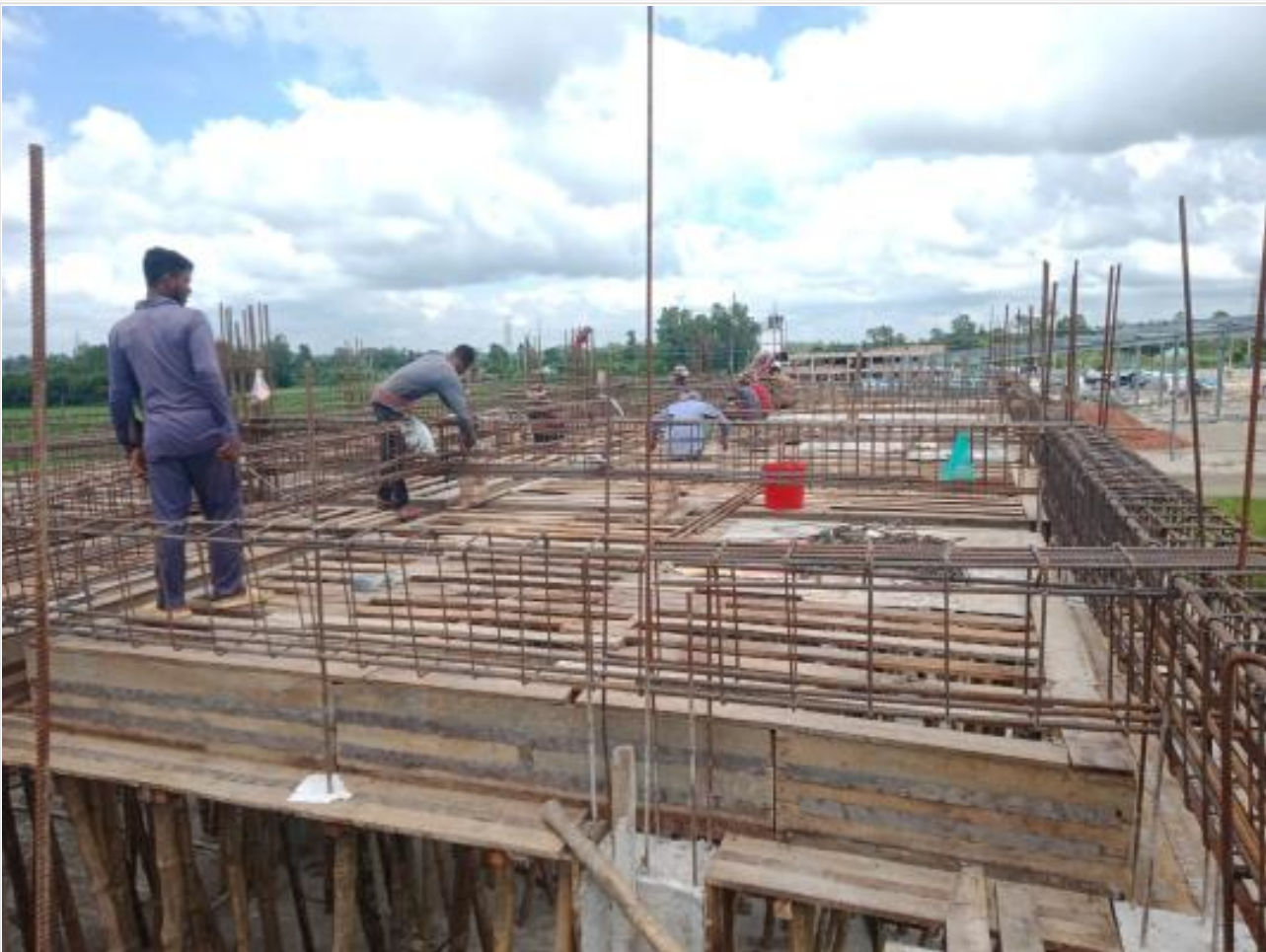
Dorm. Bldg. 2nd floor Rebar work on 07-09-23
