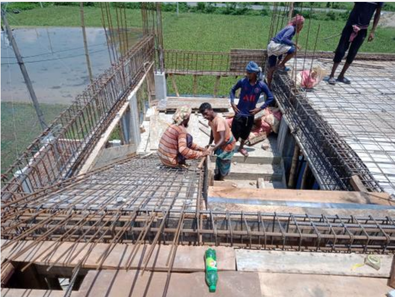
Comp. Bldg Rebar work on 31-07-23
