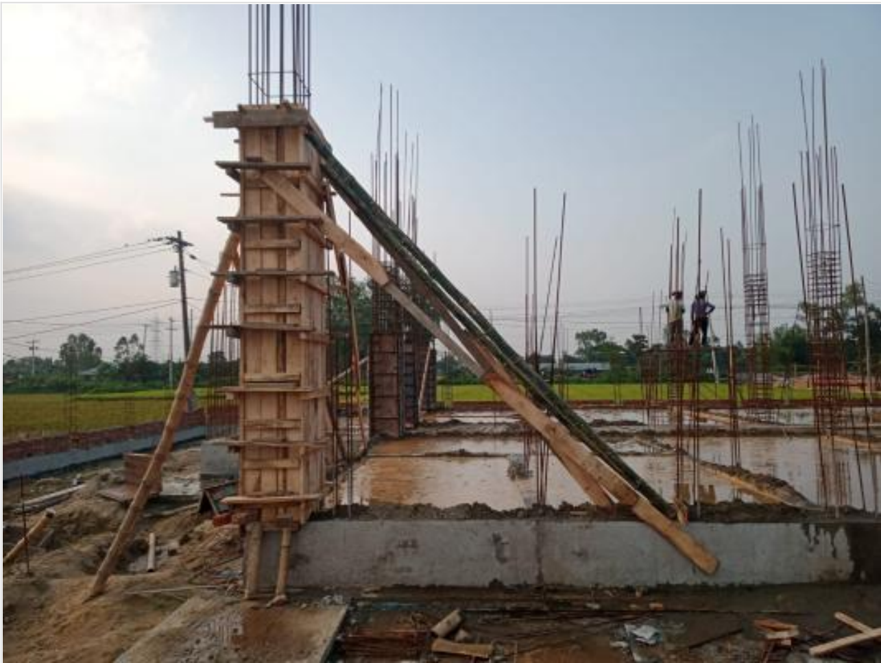
Comp. Bldg column shuttering on 26-05-23
