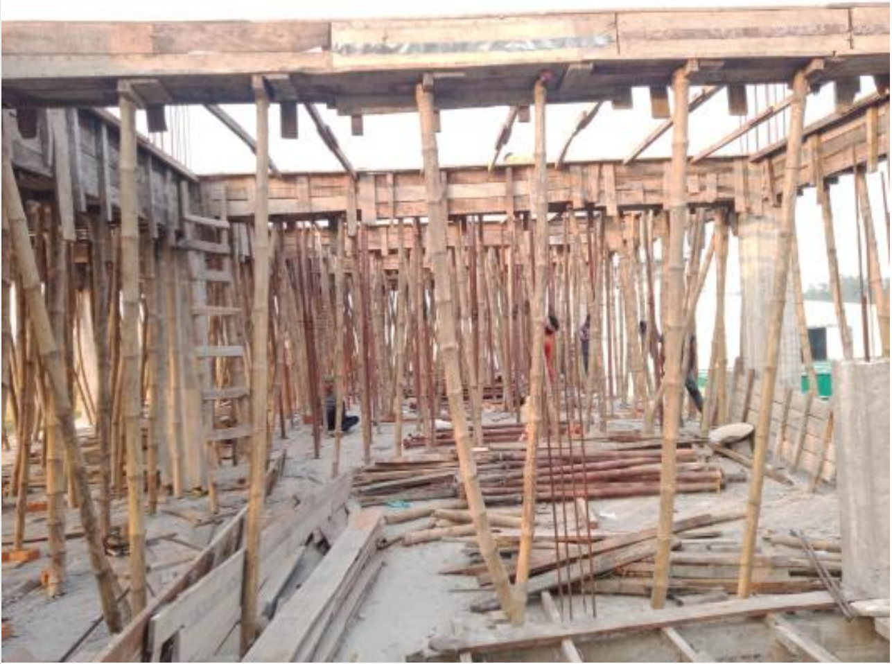
Dorm. Bldg. 3rd floor slab shuttering on 08-11-23
