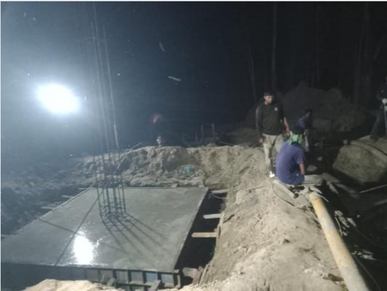
Pile Cap concreting. on 29-05-23
