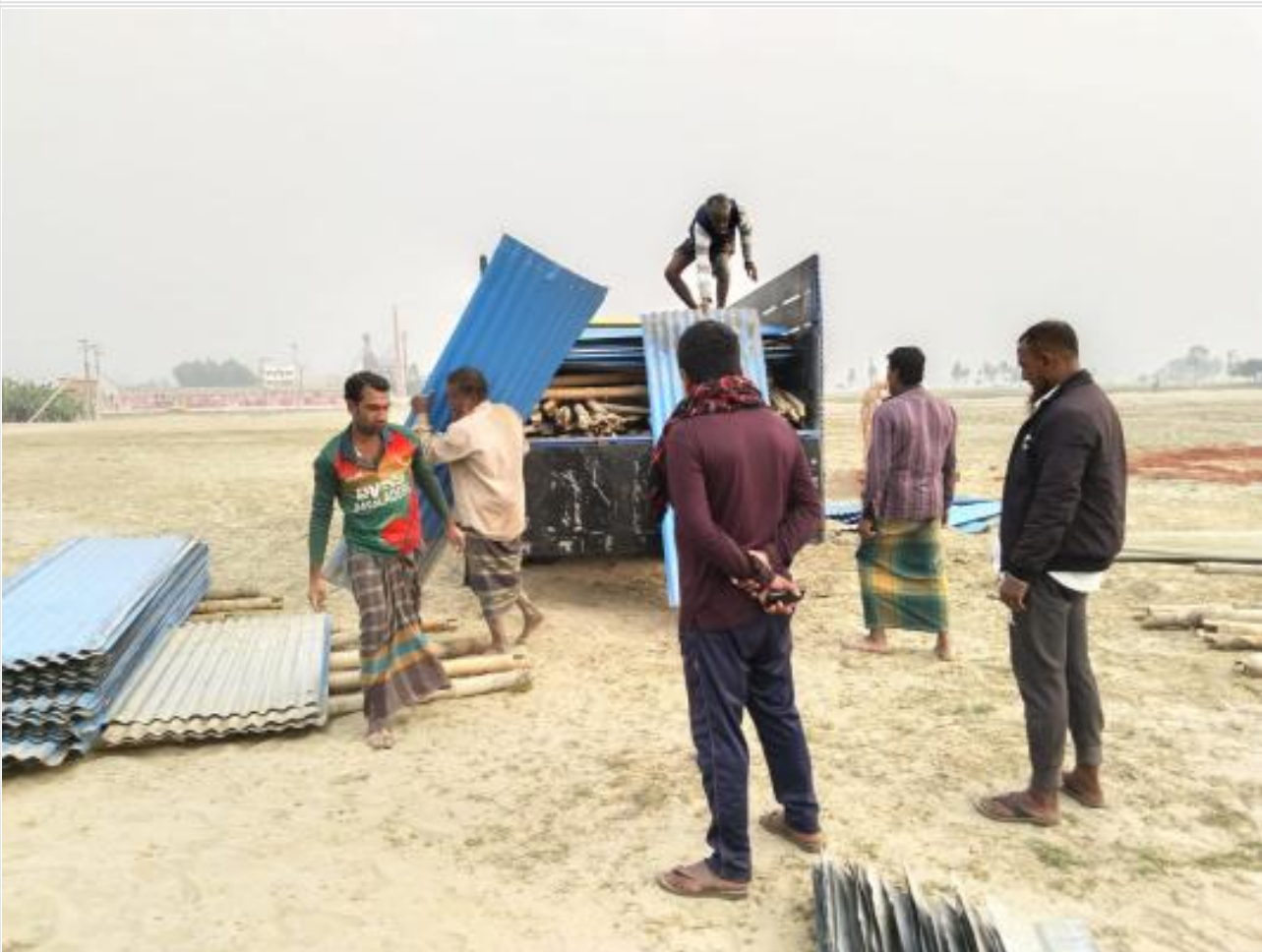
Unloading Materials on 14-01-23
