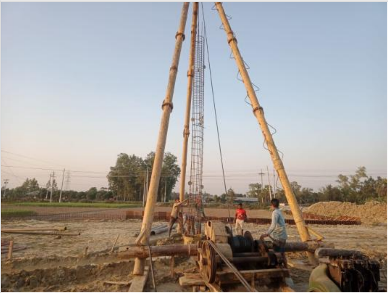
Pile boring work on 13-02-23
