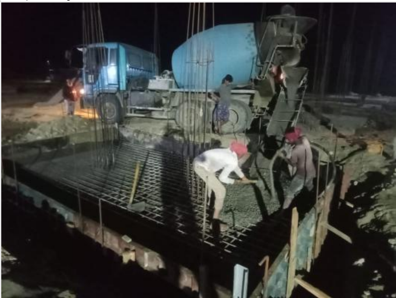
Com. Bldg. 20th pile cap casting complet on 18-04-23
