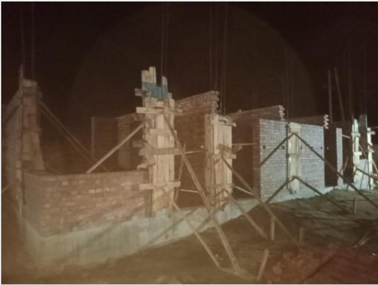
Gate House column casting on 18-06-23
