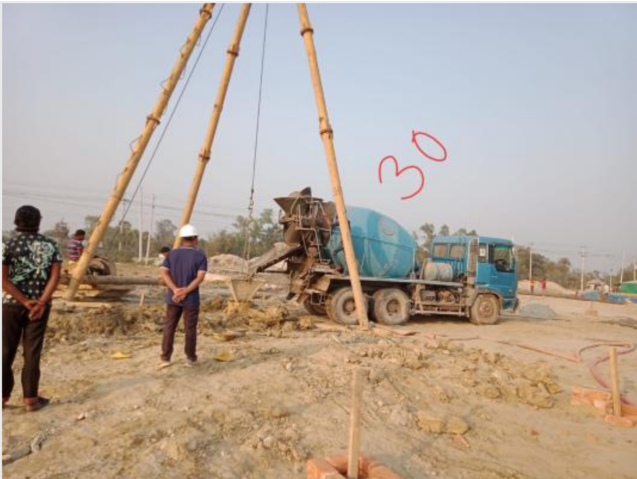
Ready mix concreting of pile on 26-02-23
