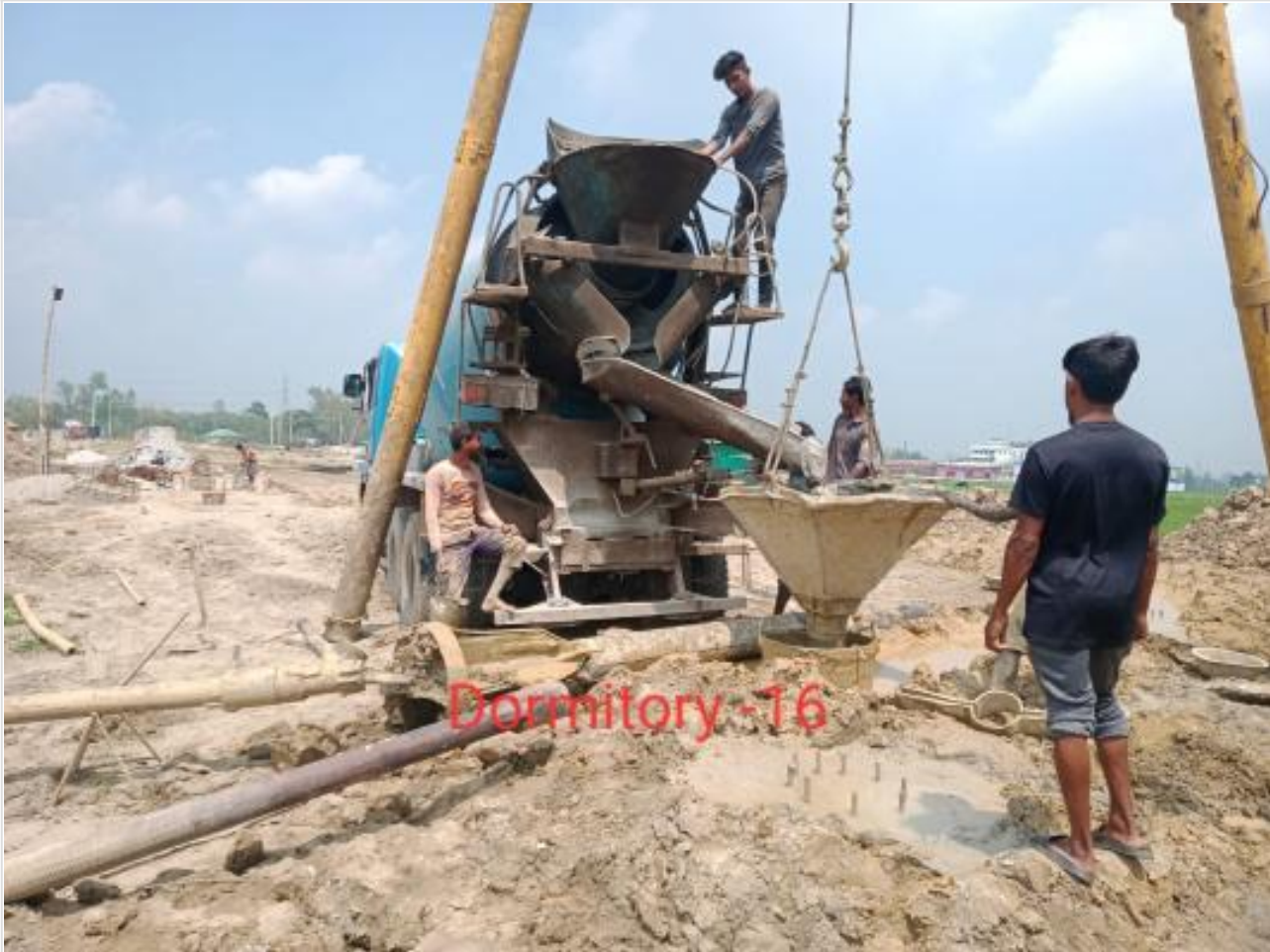
Ready mix concreting of pile on 02-04-23
