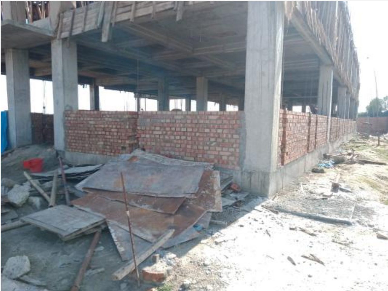
Comp. Bldg GF Brick work on 24-07-23
