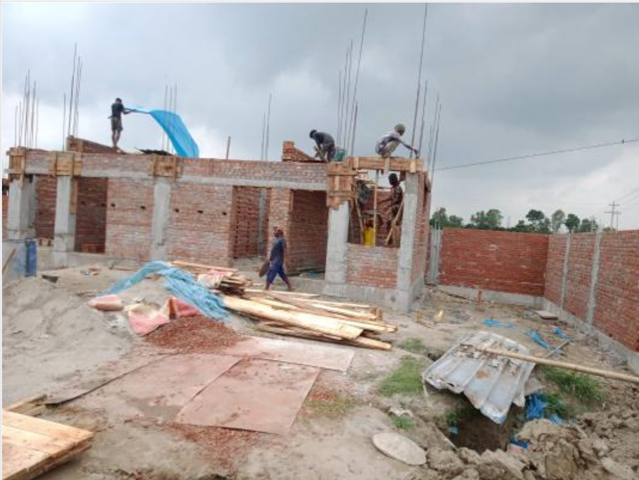
Gate House Lintel casting on 23-06-23
