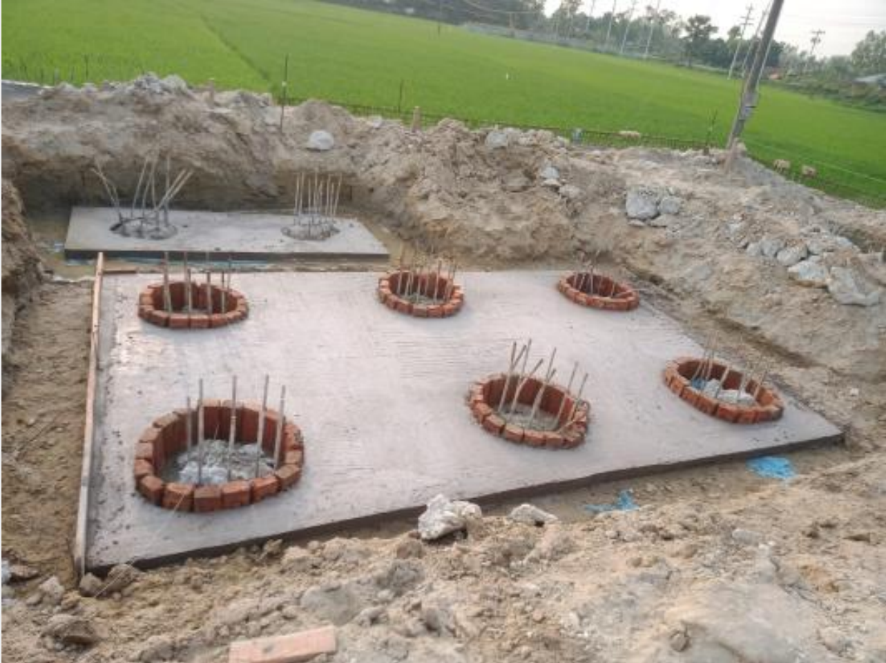
Pile cap bottom cc casting. on 04-04-23
