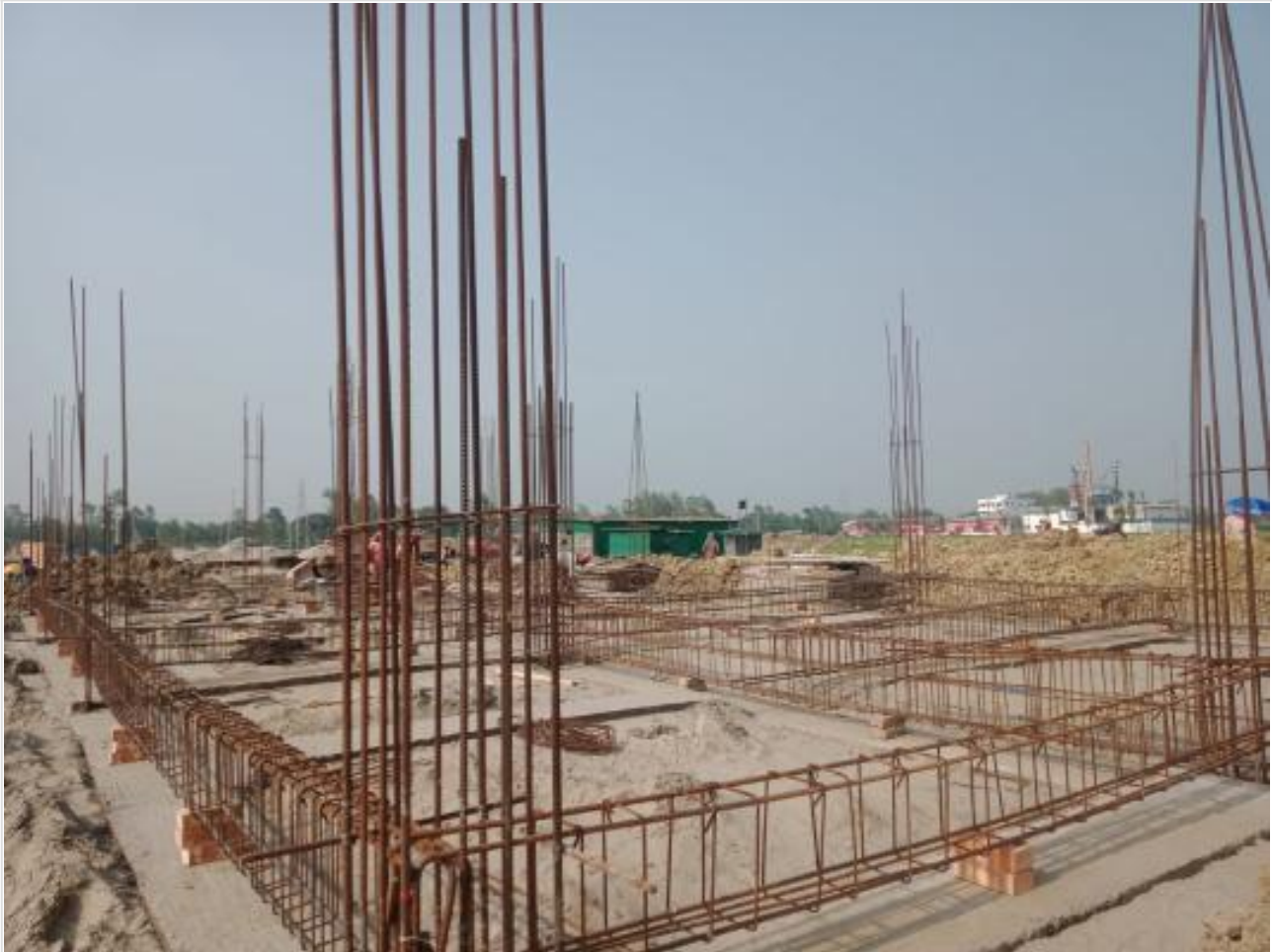
Dorm. Bldg. Rebar work for GB on 04-06-23
