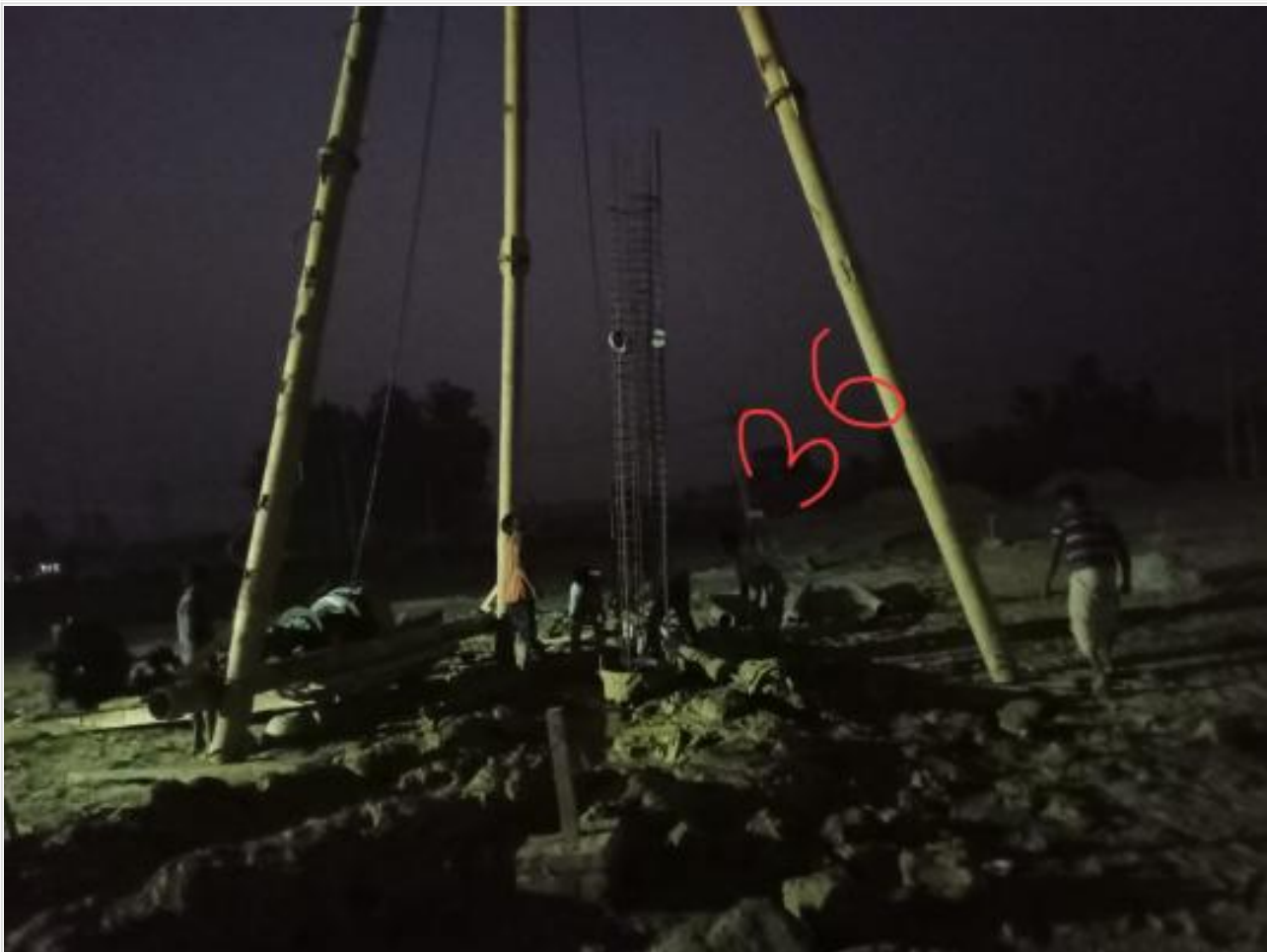
Com. Bldg. 36 Pile Boring on 28-02-23
