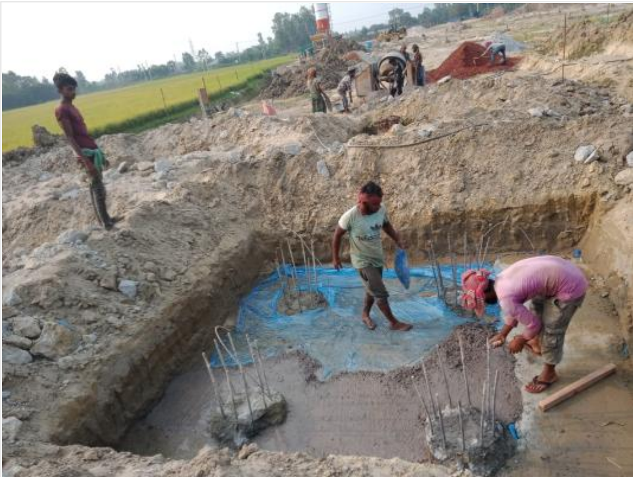
Pile cap CC work on 11-05-23
