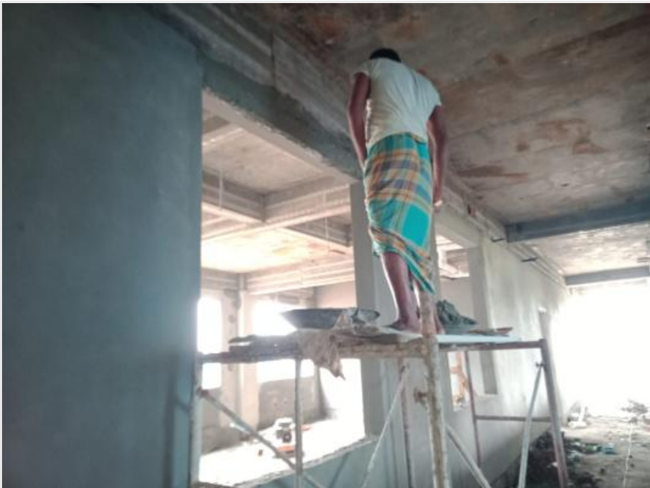
Comp. Bldg FF plastr wok on 19-09-23
