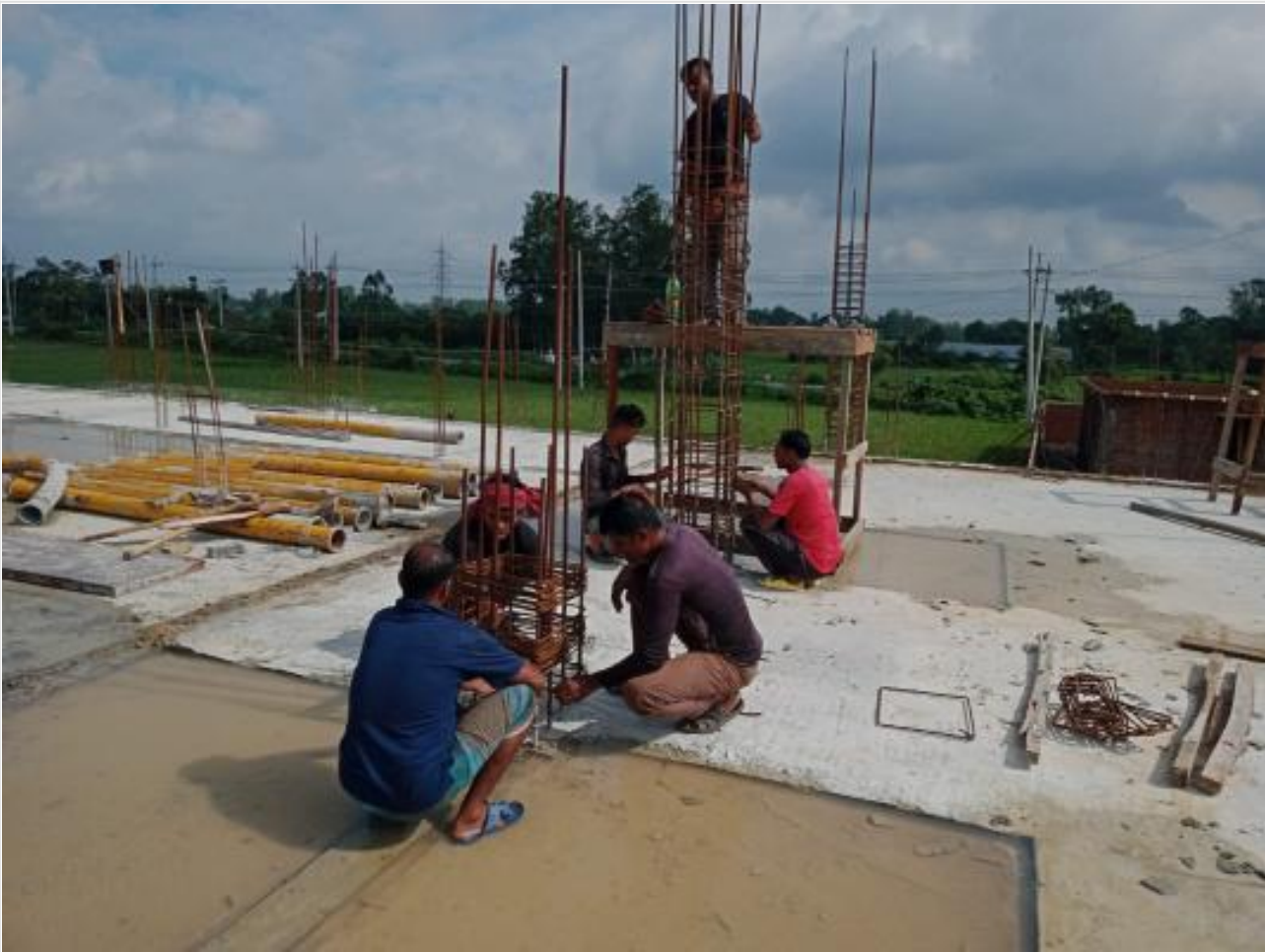
Comp. Bldg. 1st floor column rebar work on 07-07-23
