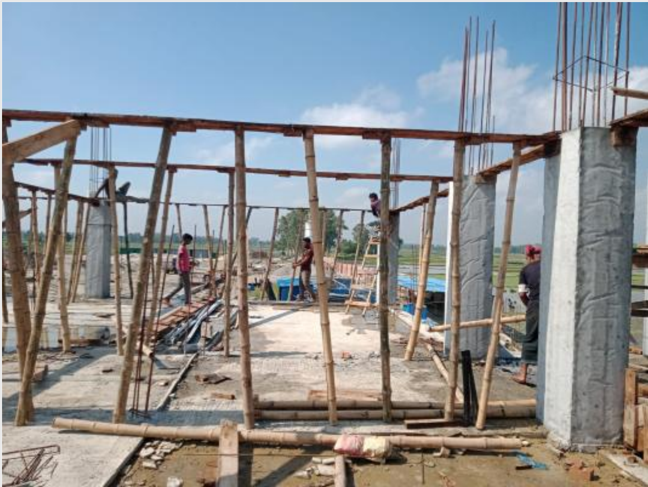
Comp. Bldg. 2nd Slab beam shuttering on 20-07-23
