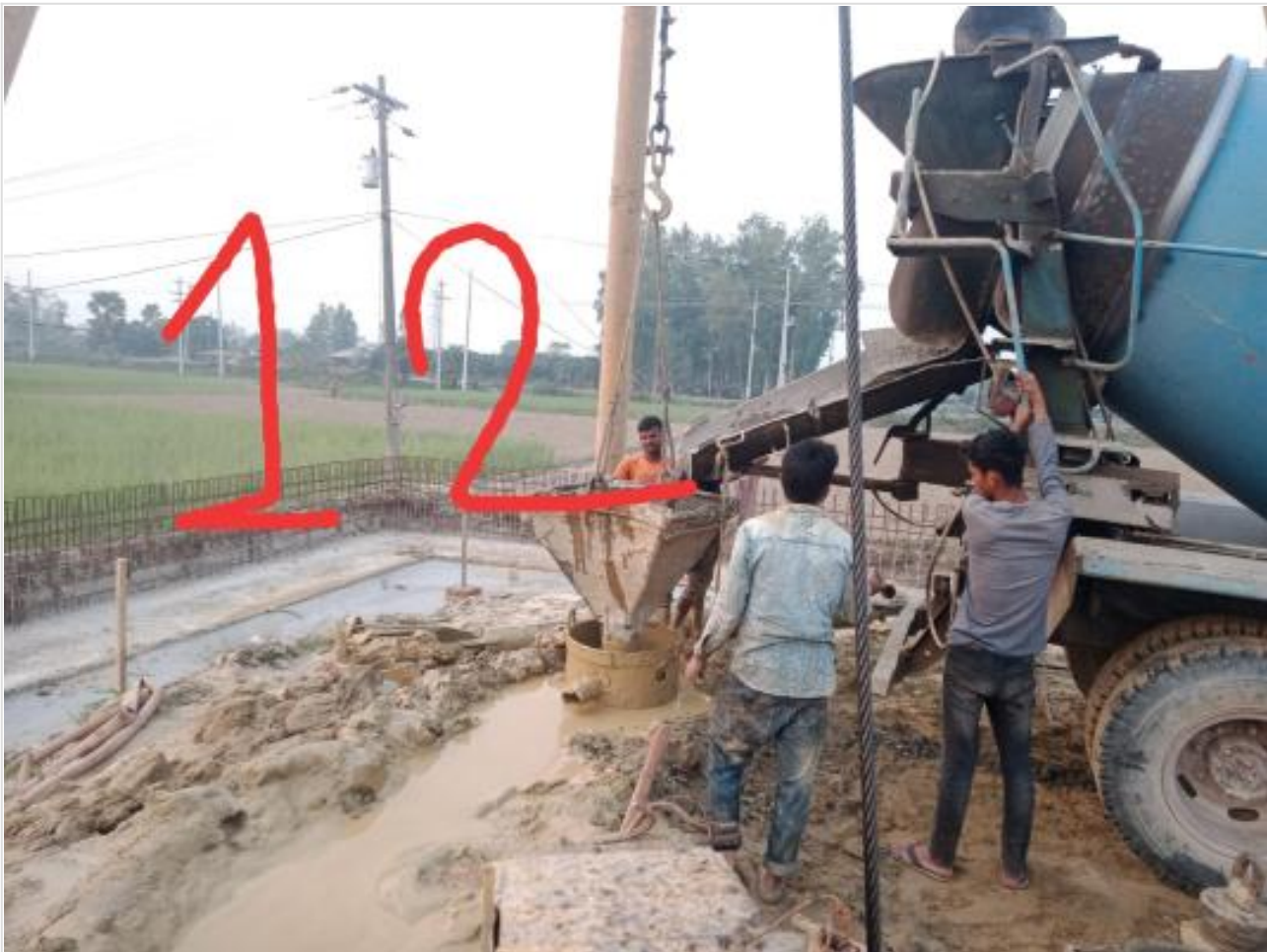
Ready mix concreting of pile on 17-02-23
