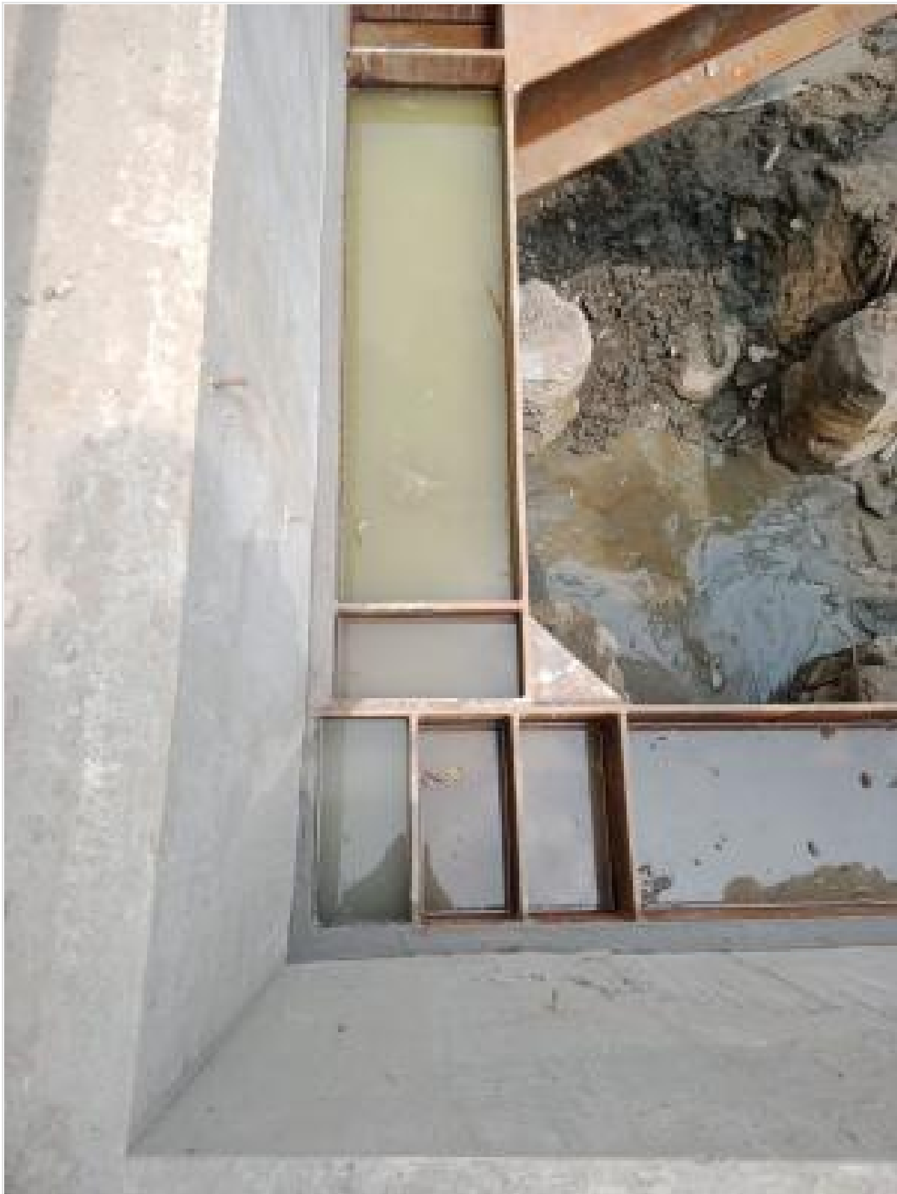
Gap filling by mortering on 02-04-22
