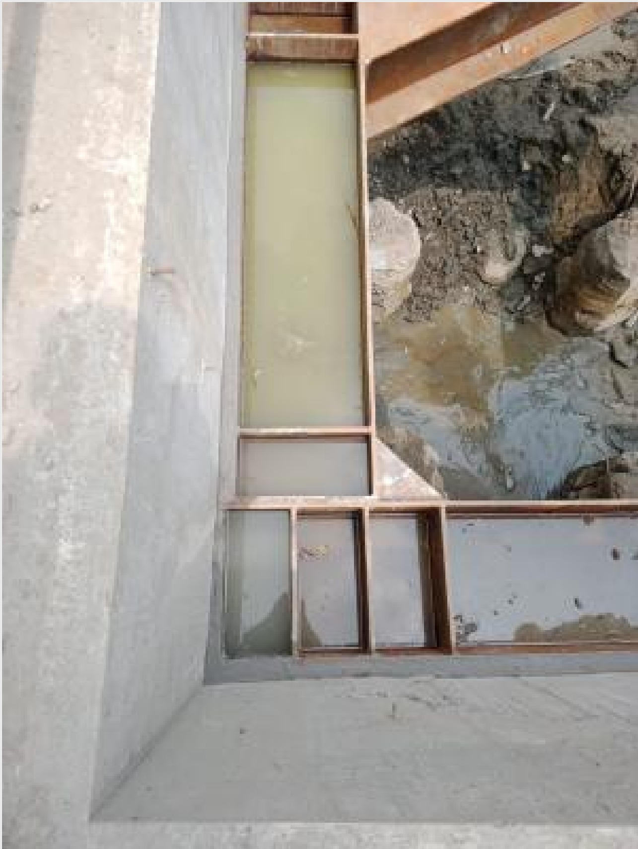
Gap filling by mortering on 02-04-22
