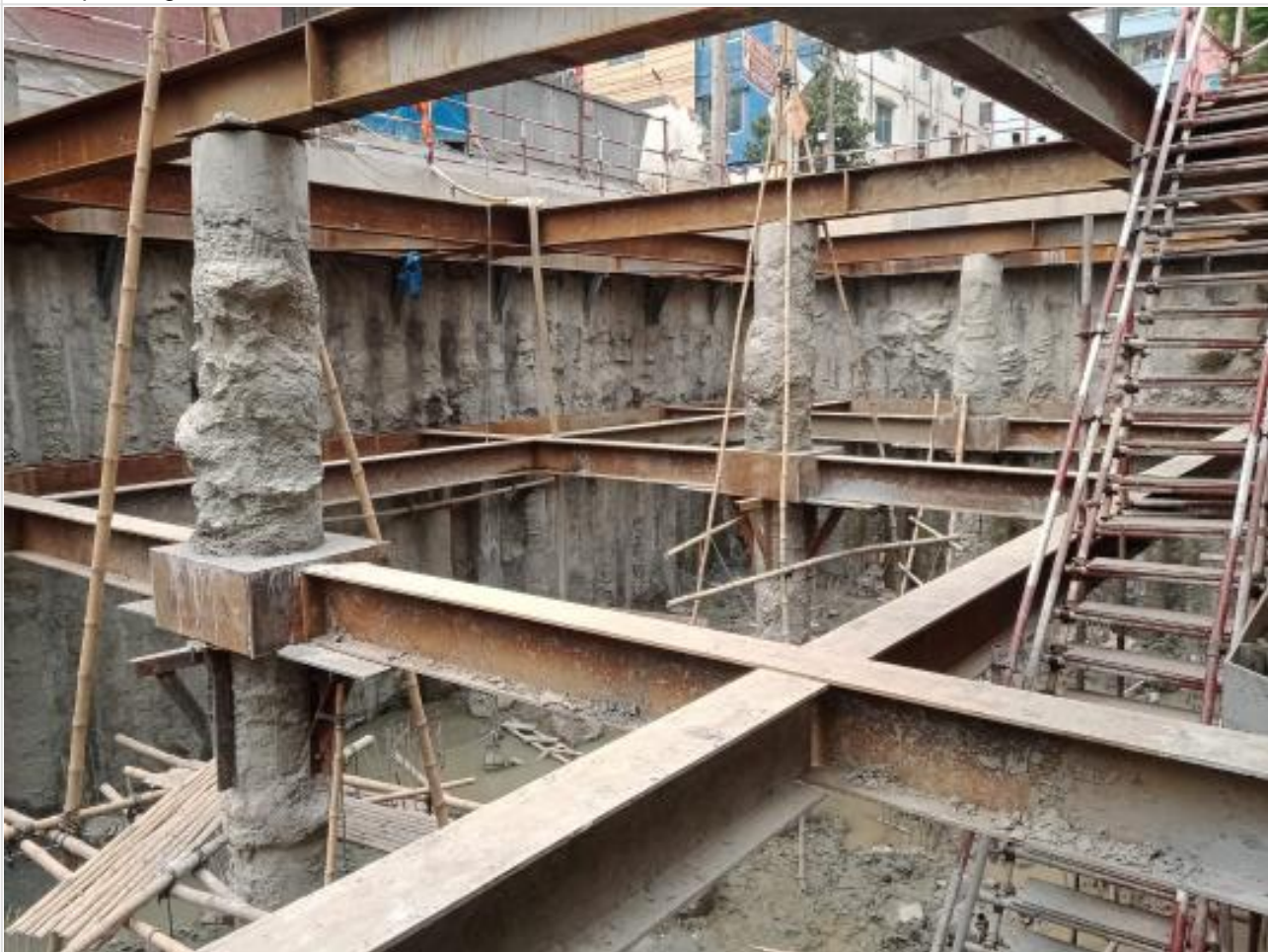
Pile gap water proofing on 30-04-22
