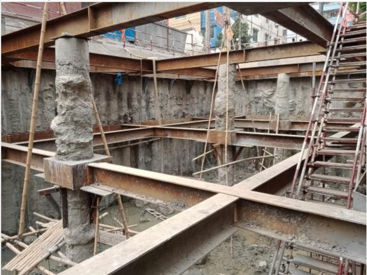
Pile gap water proofing on 30-04-22
