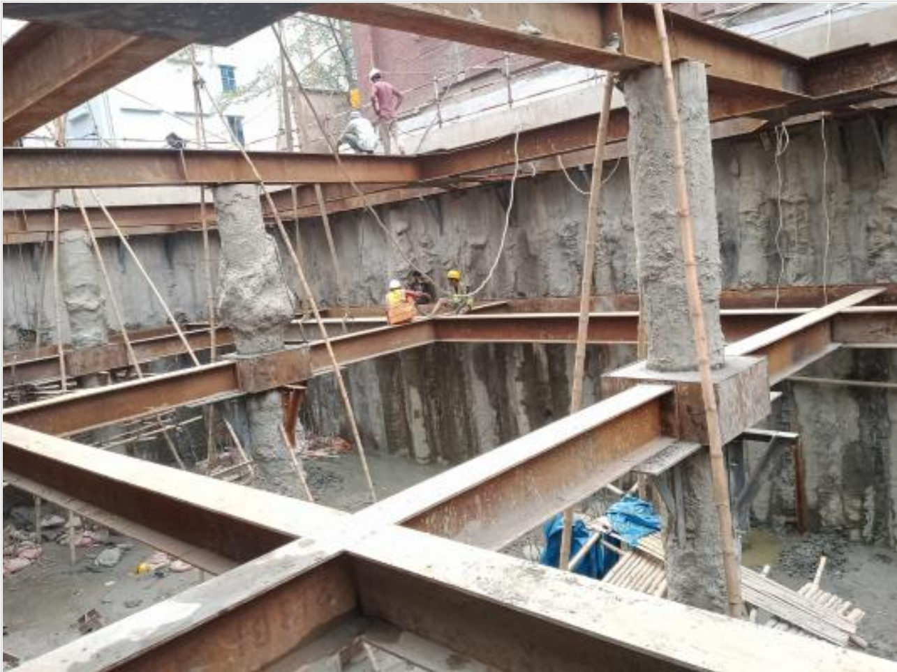
Water proofing work on 30-04-22
