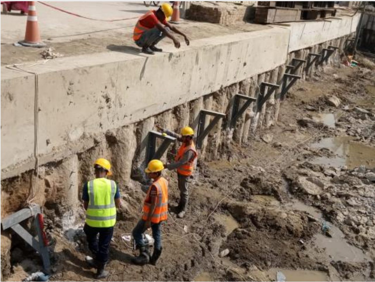
Shore pile gap filling on 16-03-22
