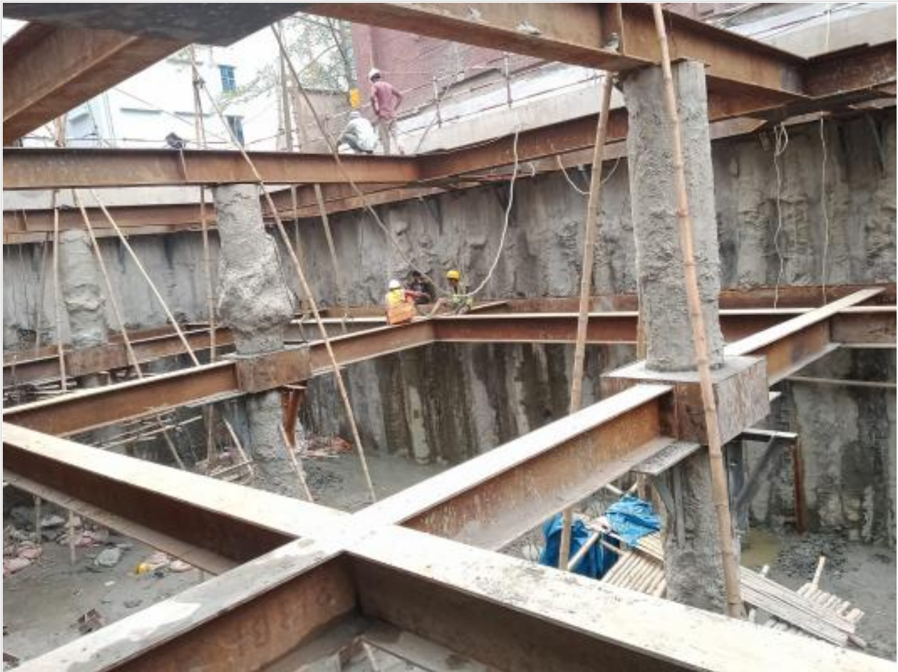
Water proofing work on 30-04-22
