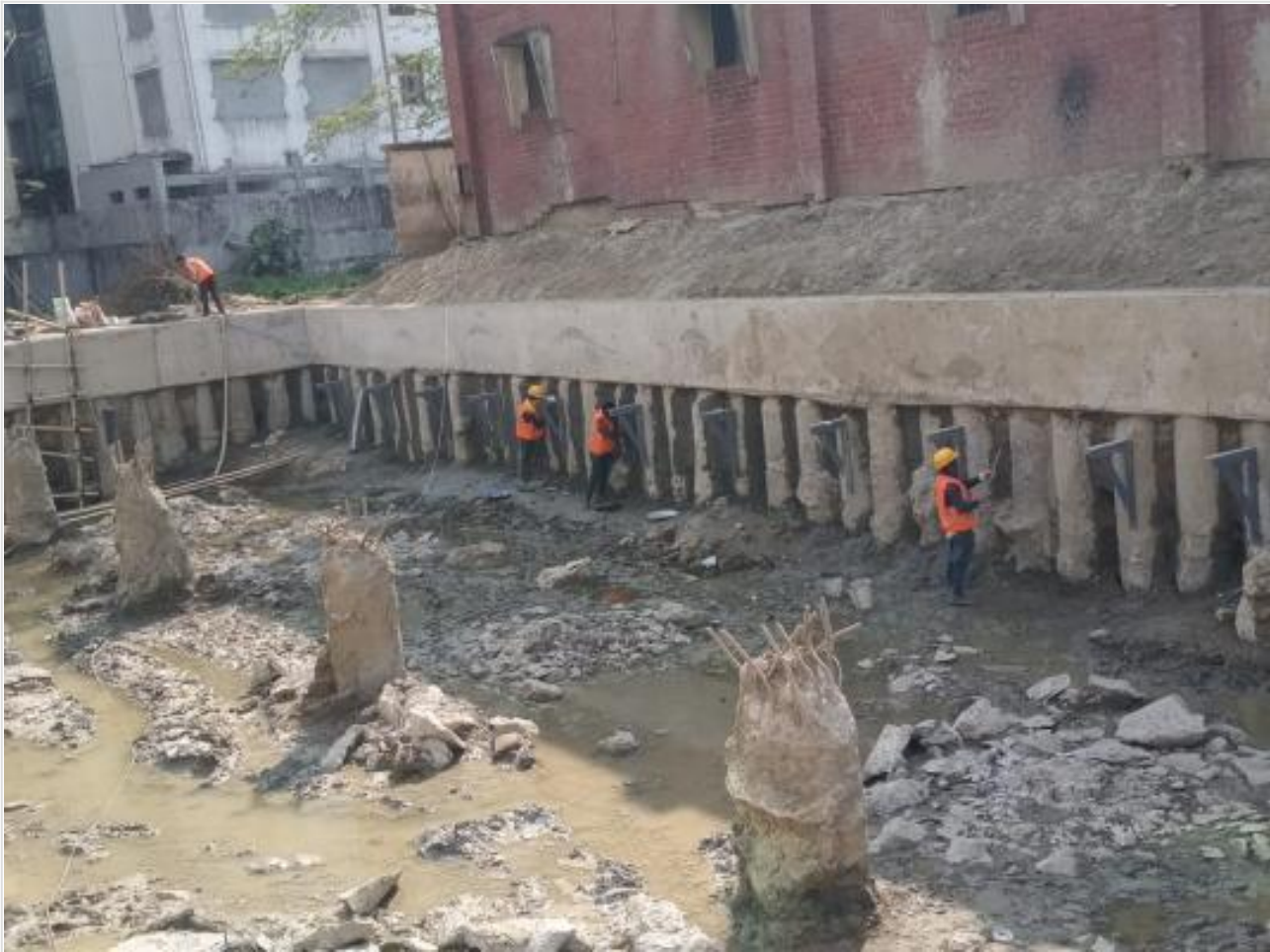
Shore pile Mortering on 16-03-22
