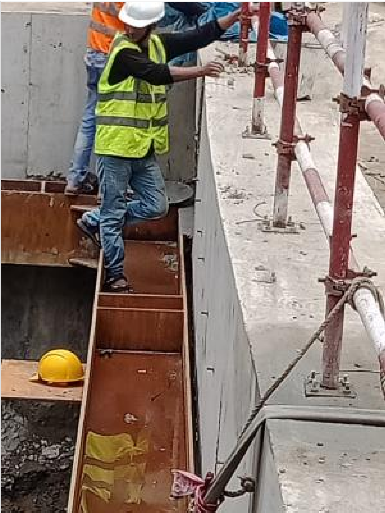
Gap filling inbetween joist and cap beam on 02-04-22
