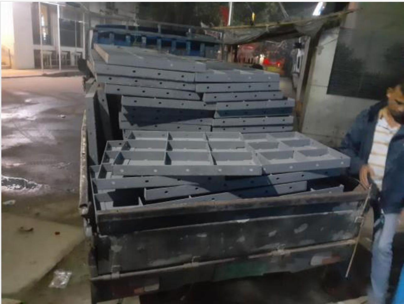
Beam Bottom shutter arrive at site parti on 22-11-21
