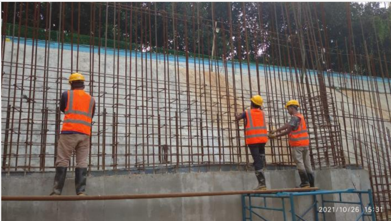
Retaining wall rebar binding on 26-10-21
