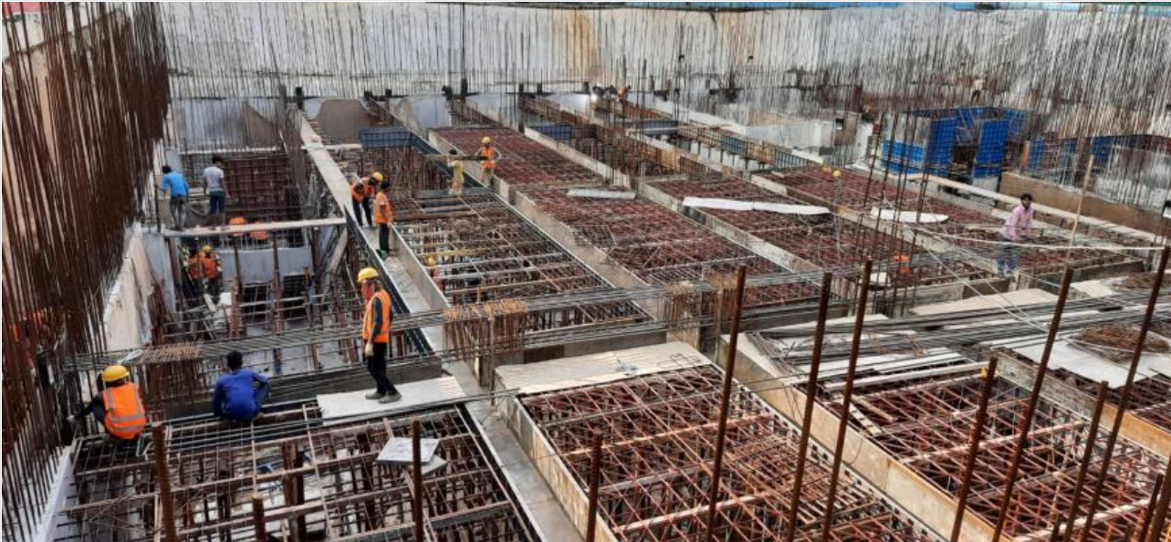
Beam rebar binding of south slab on 14-12-21
