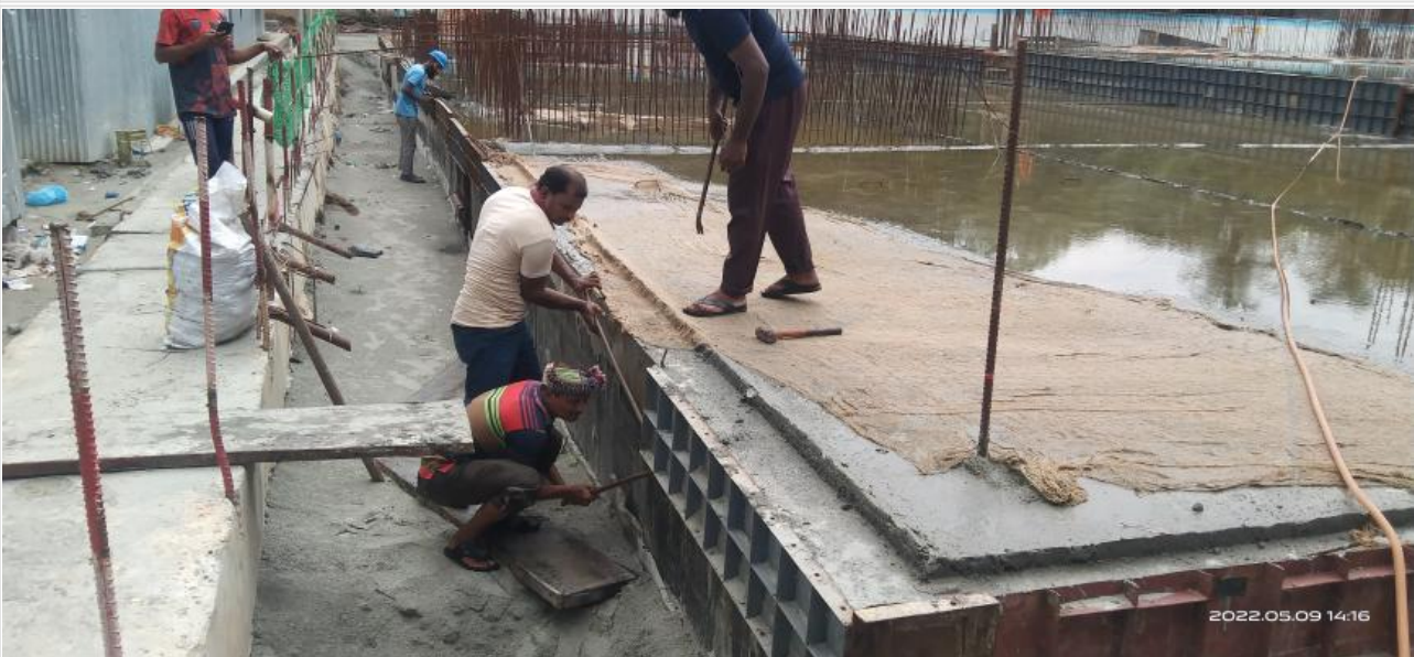
Site Shutter Remove on 09-05-22
