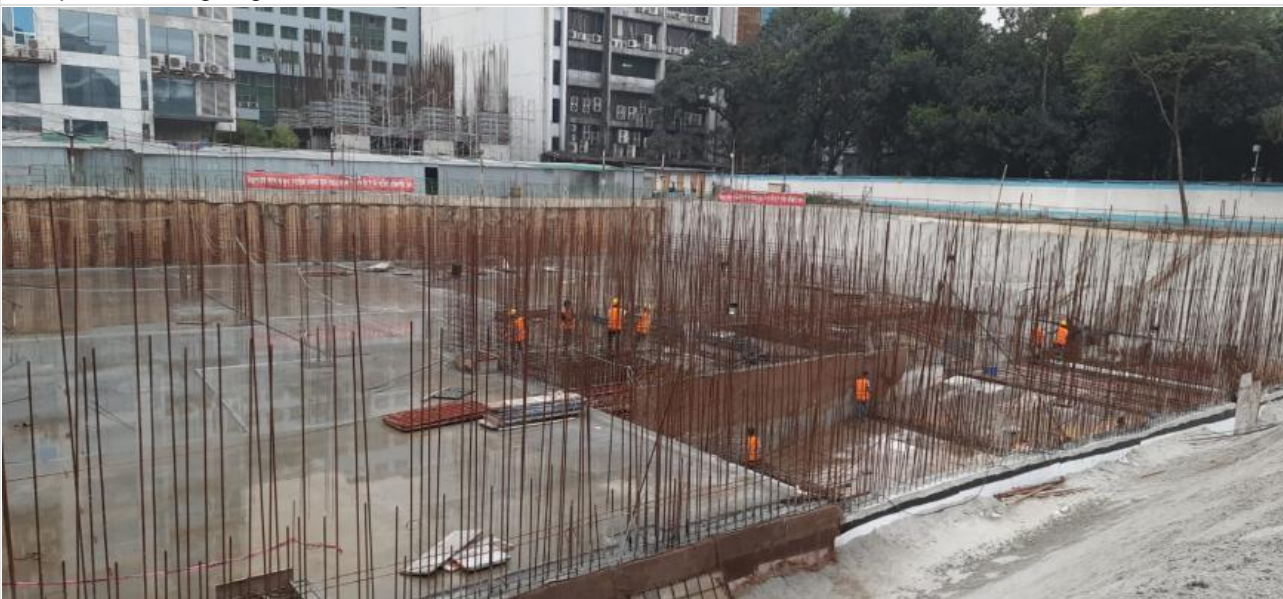
Ramp formwork going on on 26-01-22
