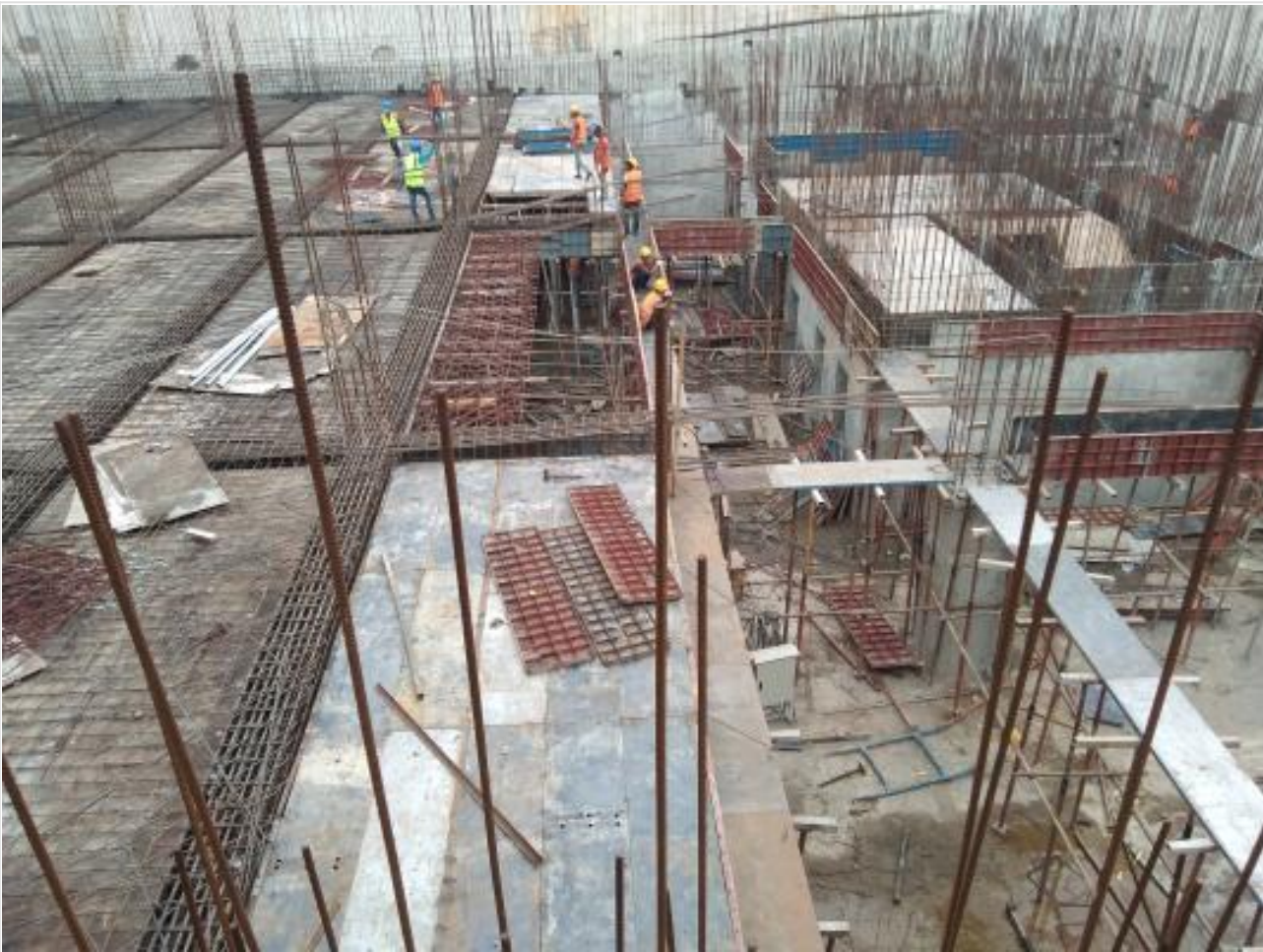
North slab shuttering on 29-12-21
