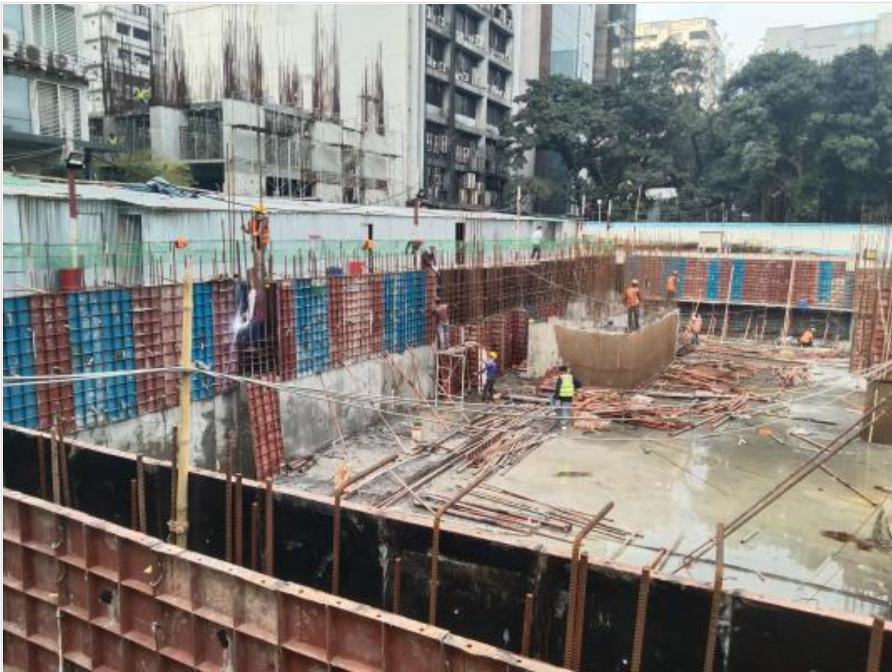
Retaining wall shuttering on 20-02-22
