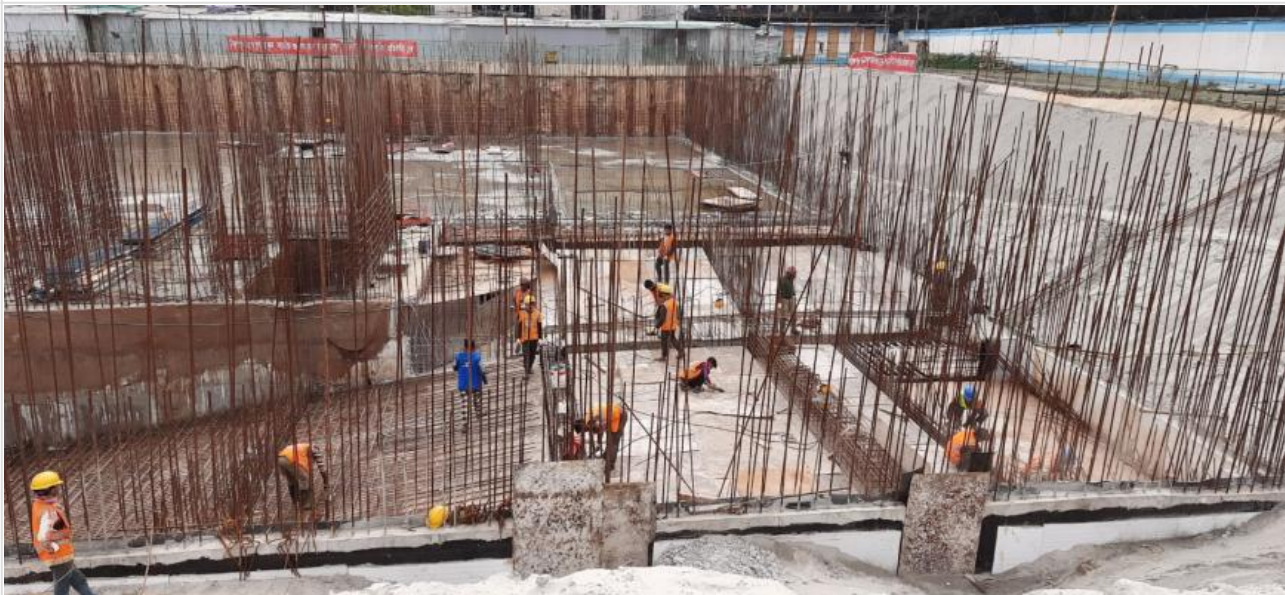
Ramp work on 28-01-22
