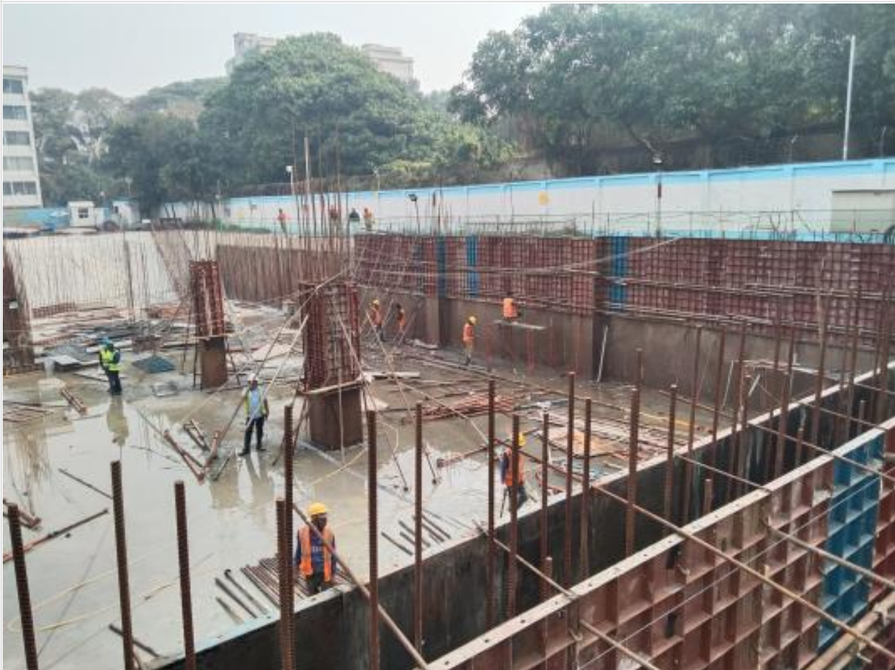
Basement-1-South Column shuttering on 23-02-22
