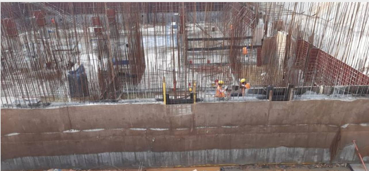
Concreting finish at 12:45PM on 19-11-2021
