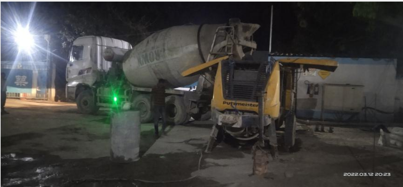
Ready mix on 13-03-22
