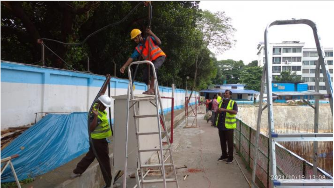
Service cable line work on 19-10-21
