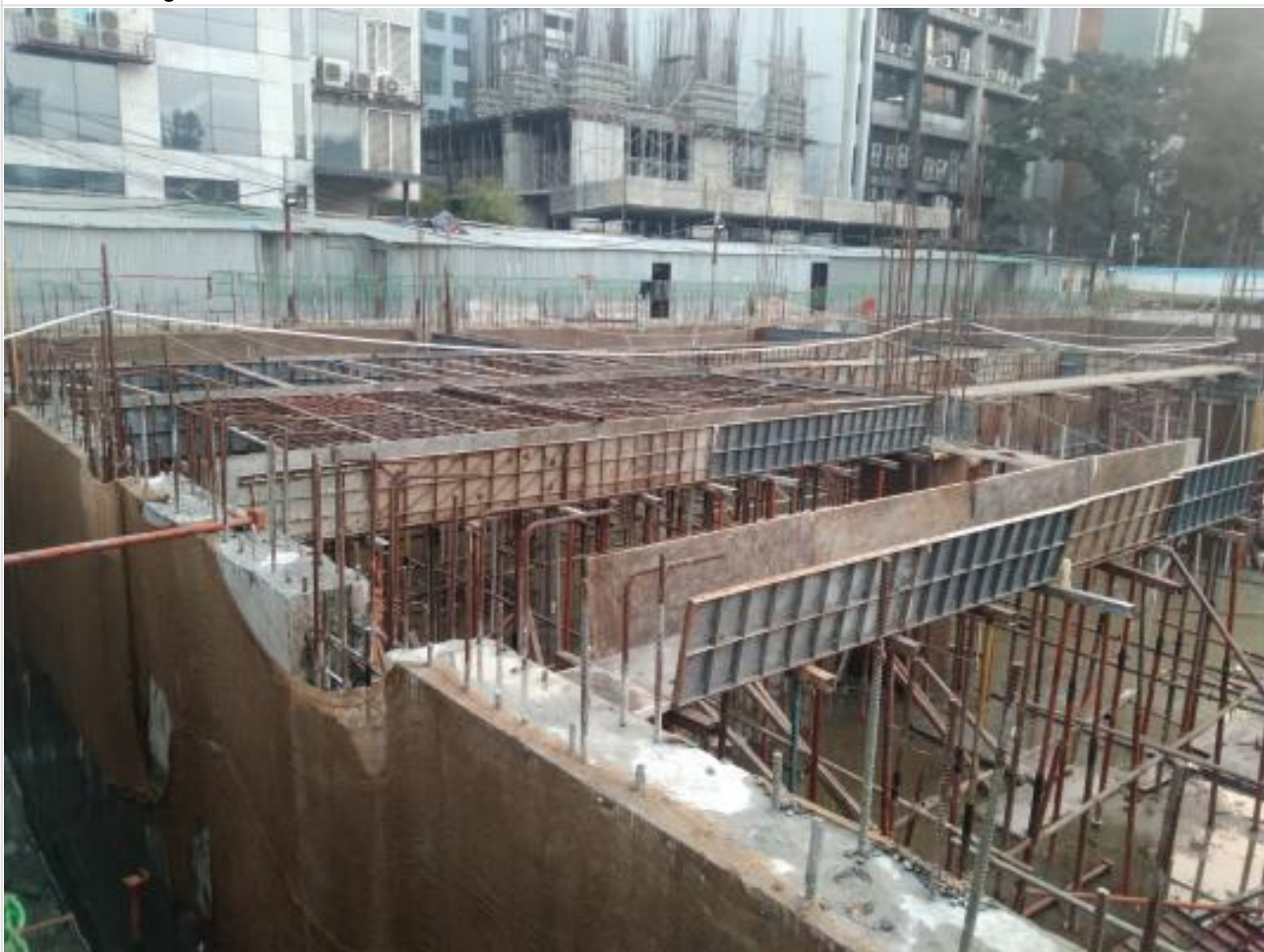
South GF slab shutter on 07-03-22
