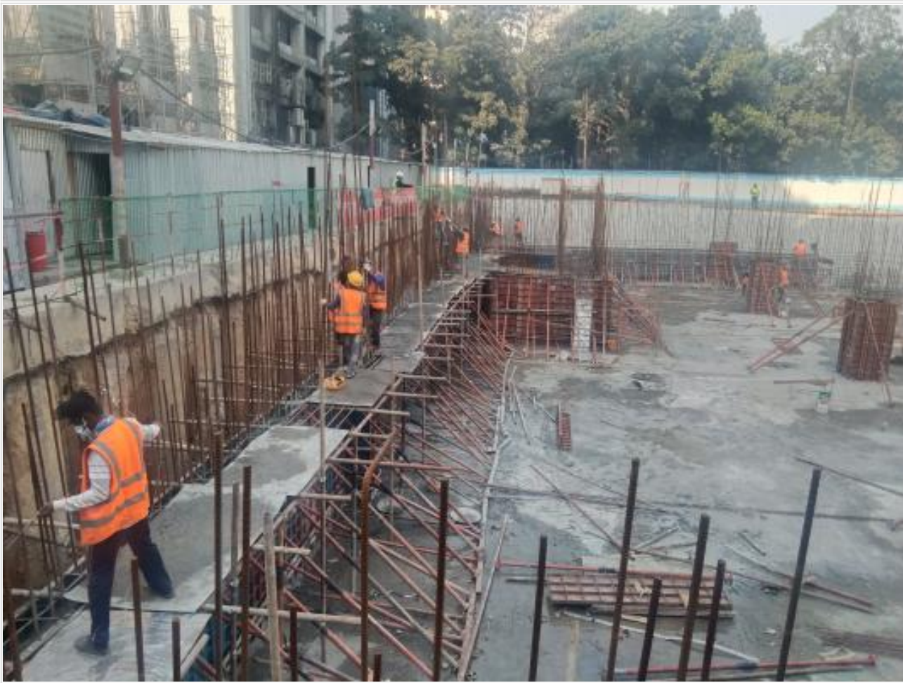
Basement-1-South retaining wall 2nd lift on 16-02-22
