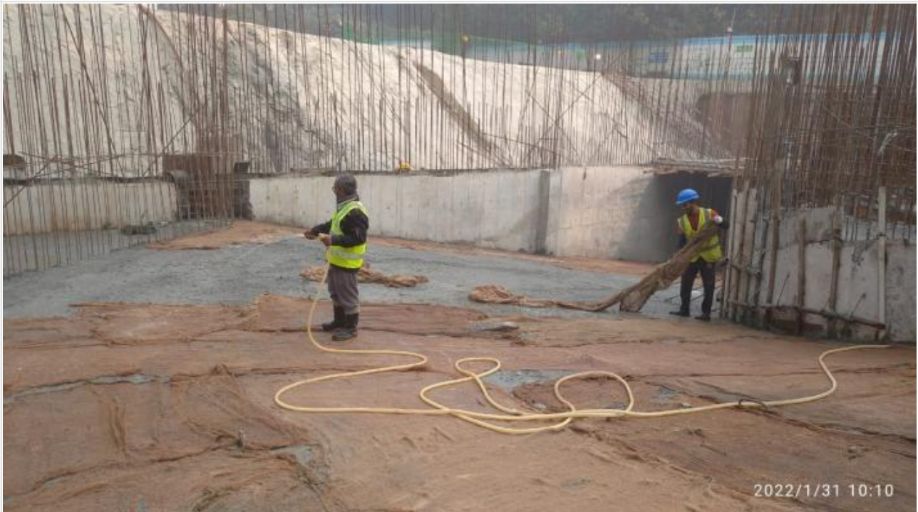
Ramp Curing work on 31-01-22
