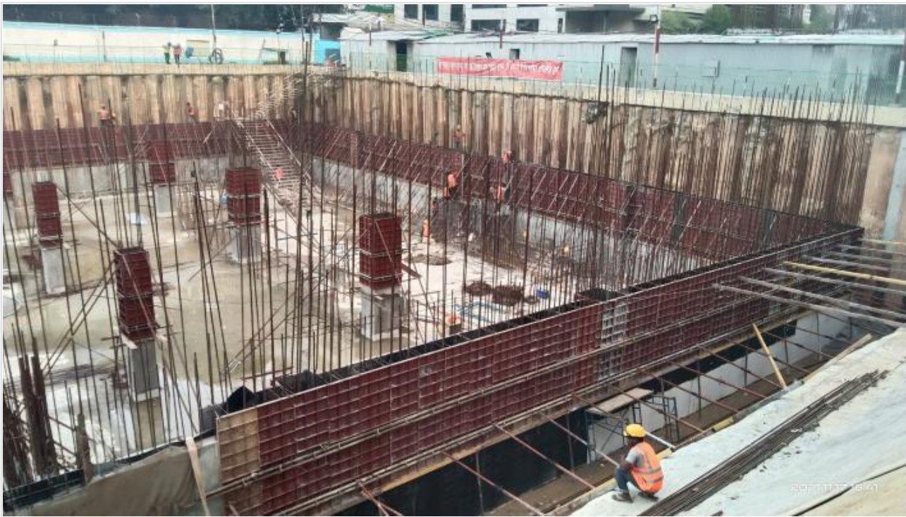
South retaining wall on 17-11-21
