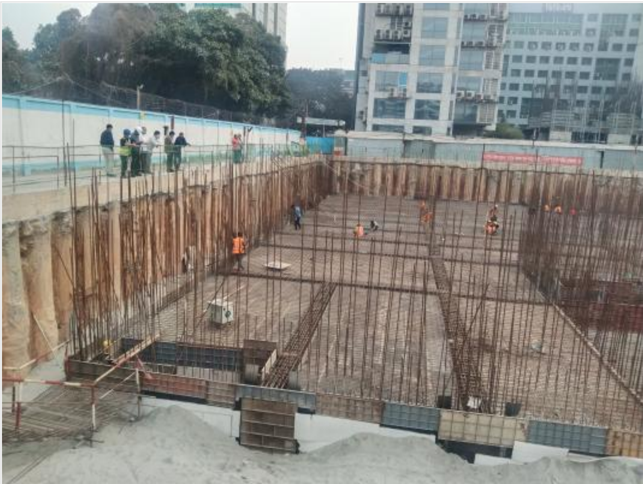
North south slab work on 11-01-22
