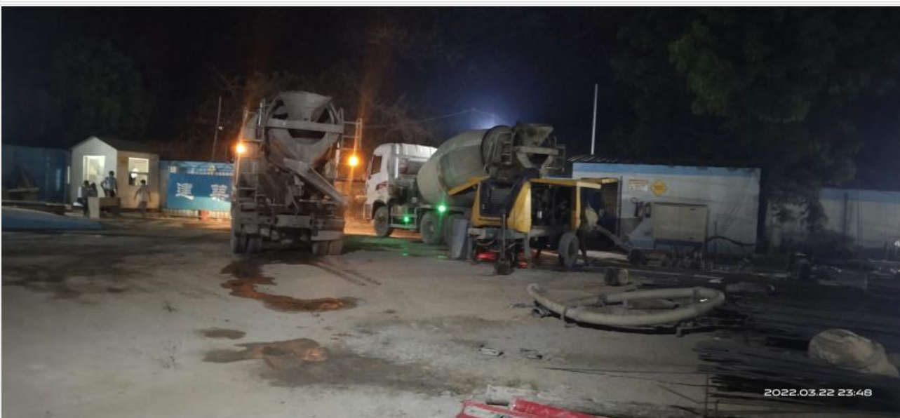
Ready mix on 22-03-22
