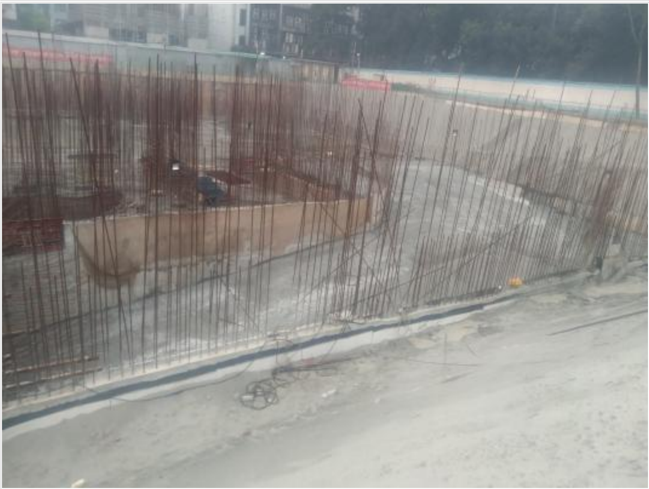
Ramp concreted on 31-01-22
