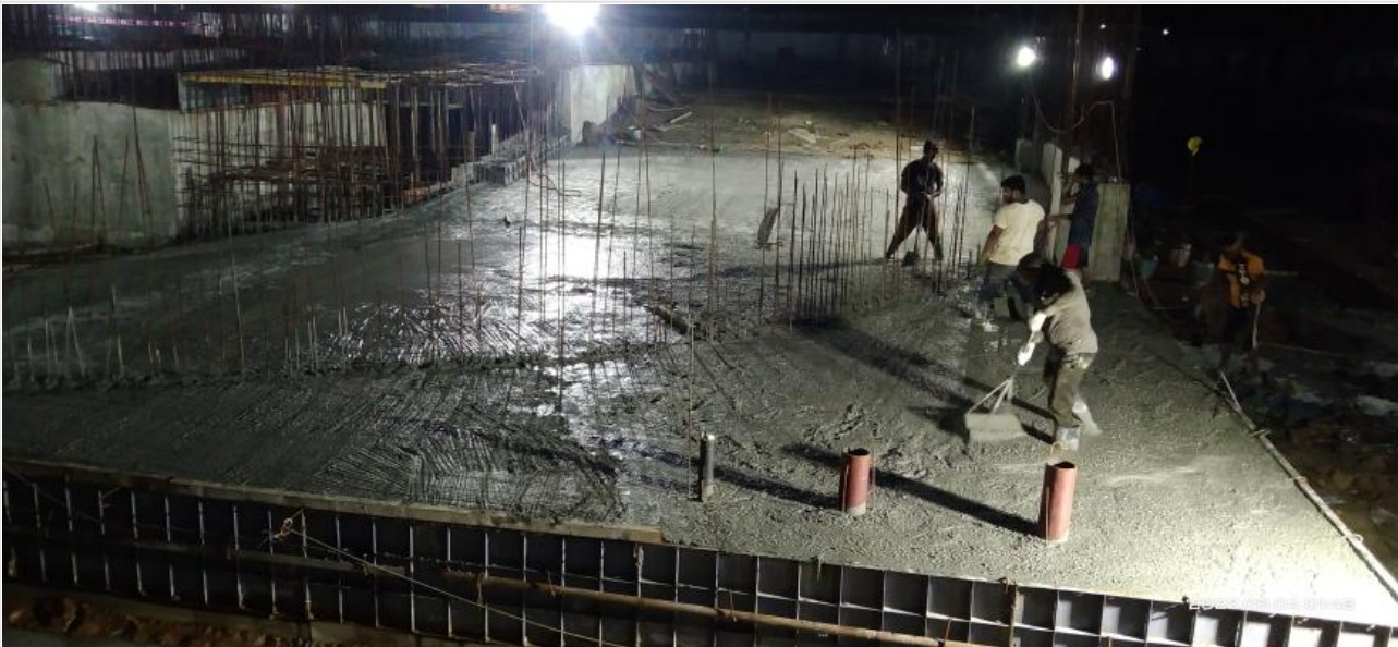
Ready mix concreting on 03-06-22
