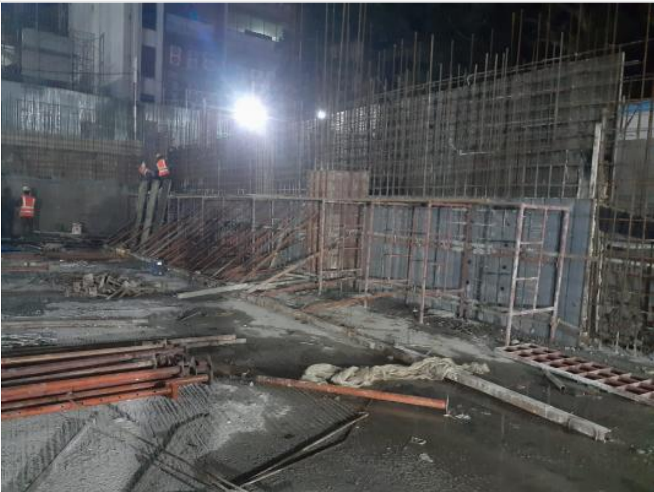
Shuttering work on 18-02-22
