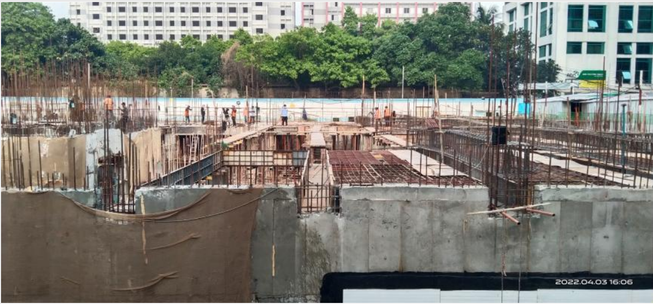
Work progress on 03-04-22
