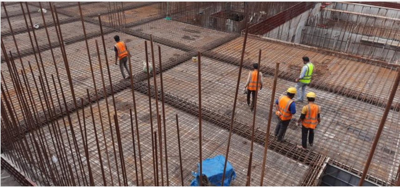
Slab levelling on 12-01-22
