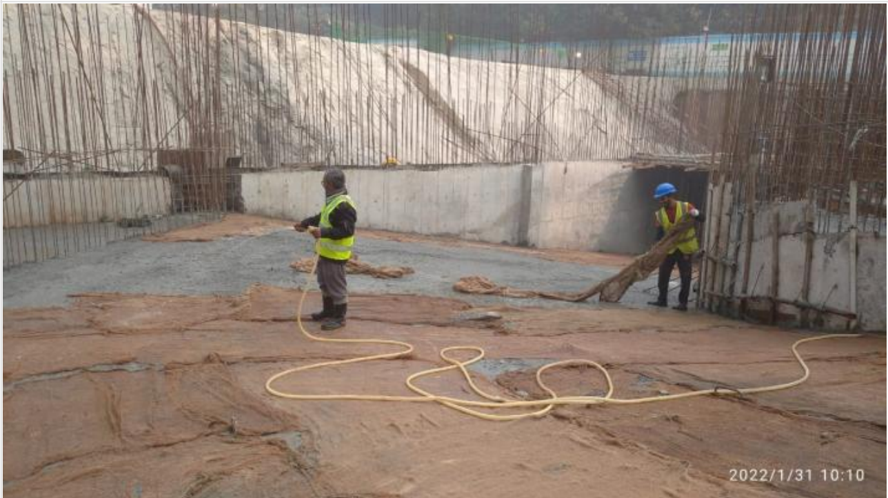
Ramp Curing work on 31-01-22
