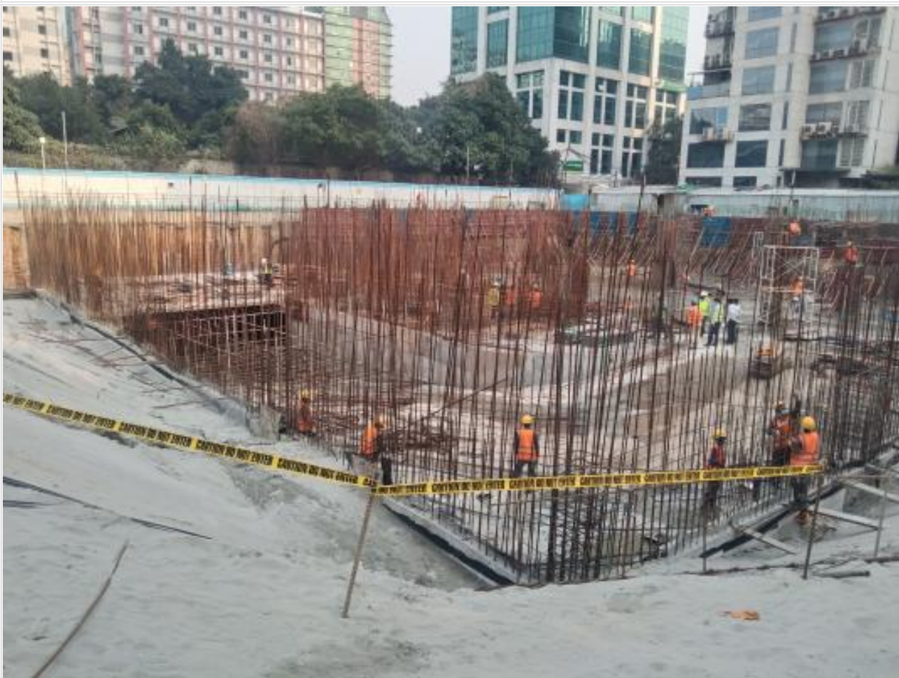
B-1-North retaining wall rebar work on 28-02-22
