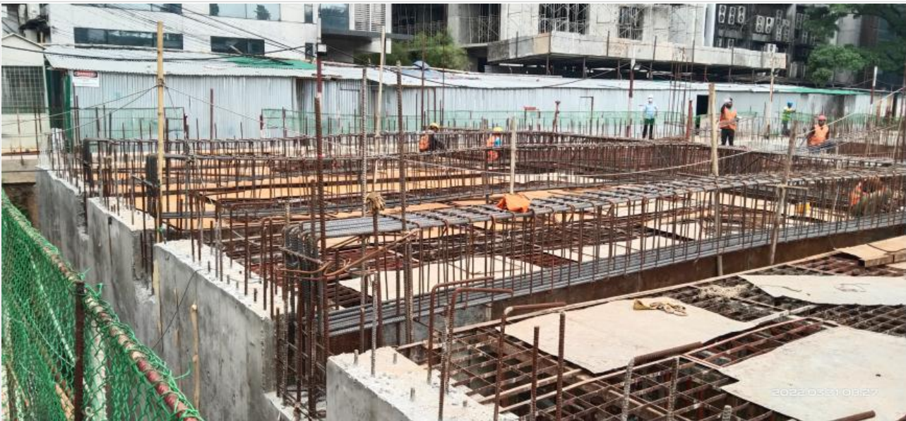
Gr.Floor Slab shuttering and rod binding on 31-03-22
