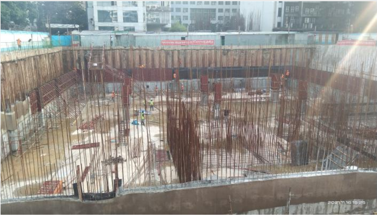
South Retaining on 16-11-21
