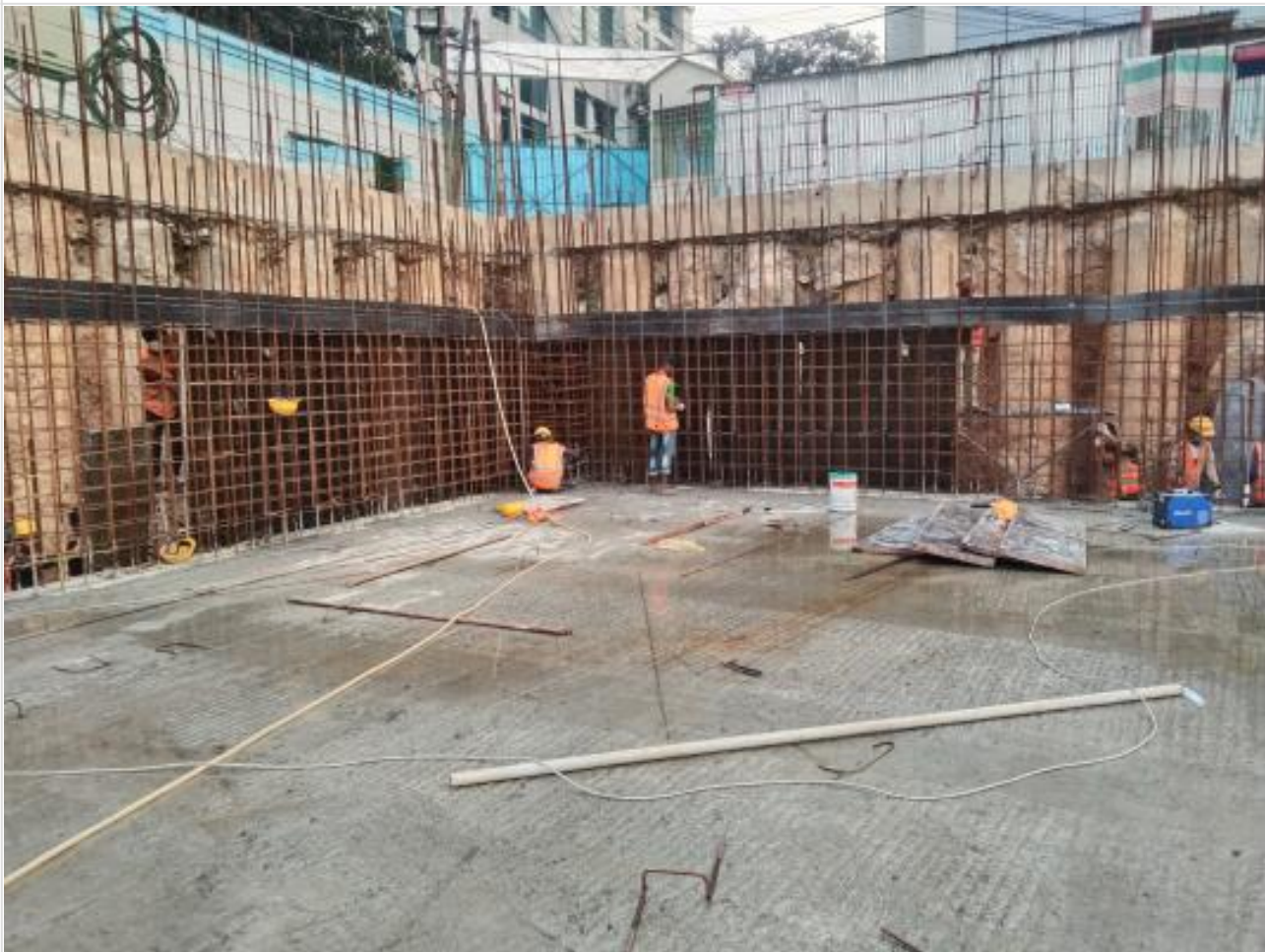
South Retaining wall shuttering on 09-02-22
