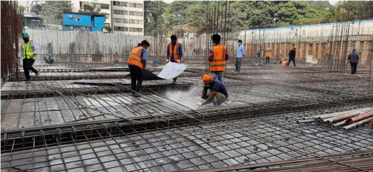
North slab work on 04-01-22
