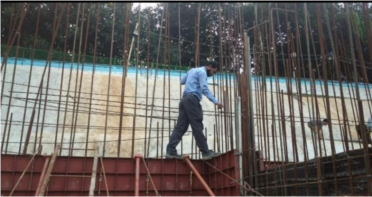
North Retaining wall inspection on 04-11-21
