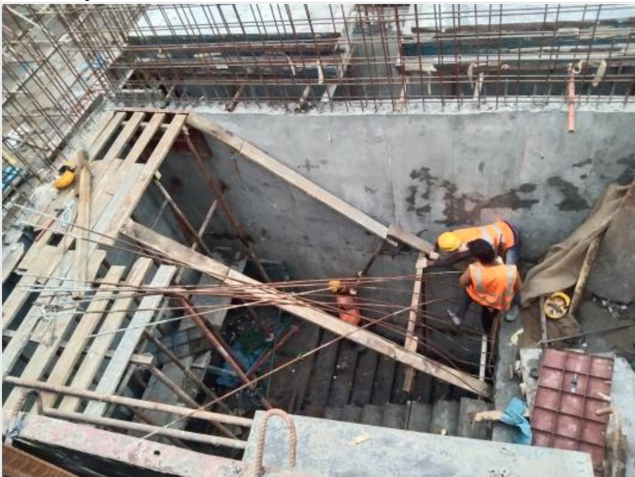
South stair work on 22-02-22
