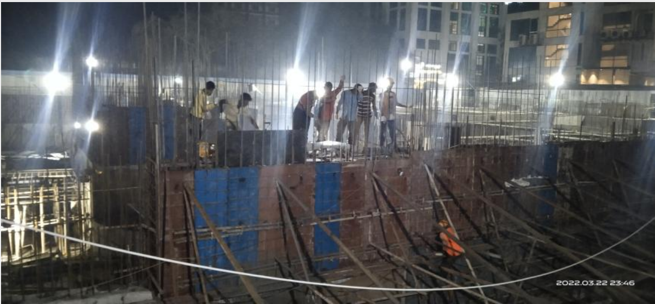
Ready mix casting on 22-03-22
