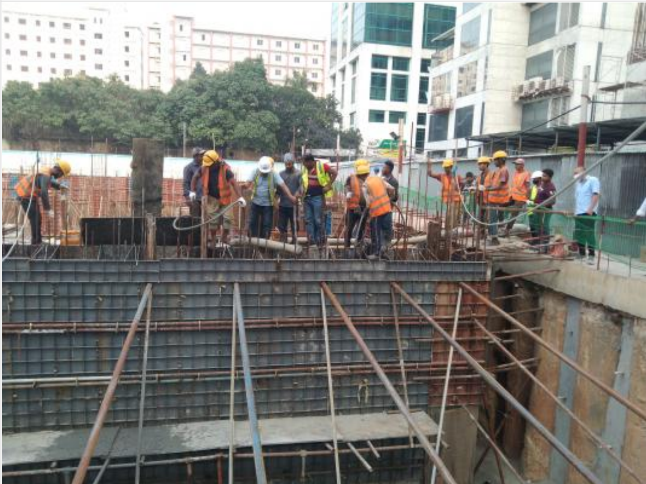
B-1-South 2nd Retaining wall concreting on 26-02-22
