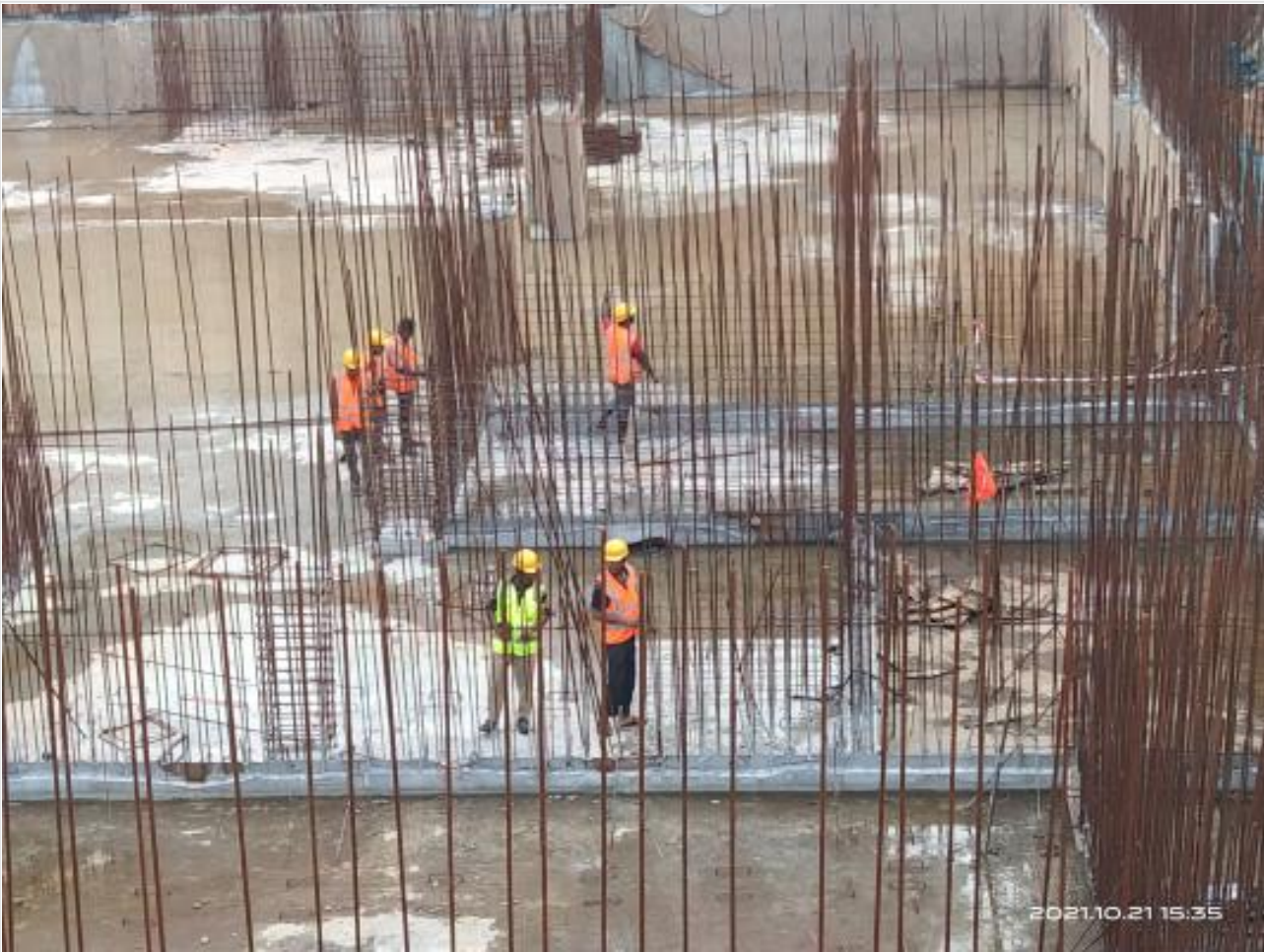
Rebar work on 21-10-21
