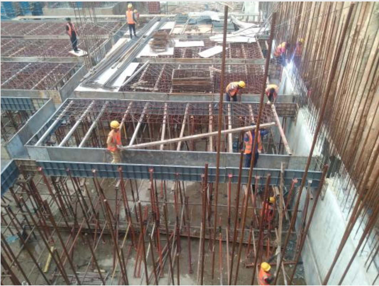
B1 south slab shuttering on 13-12-21
