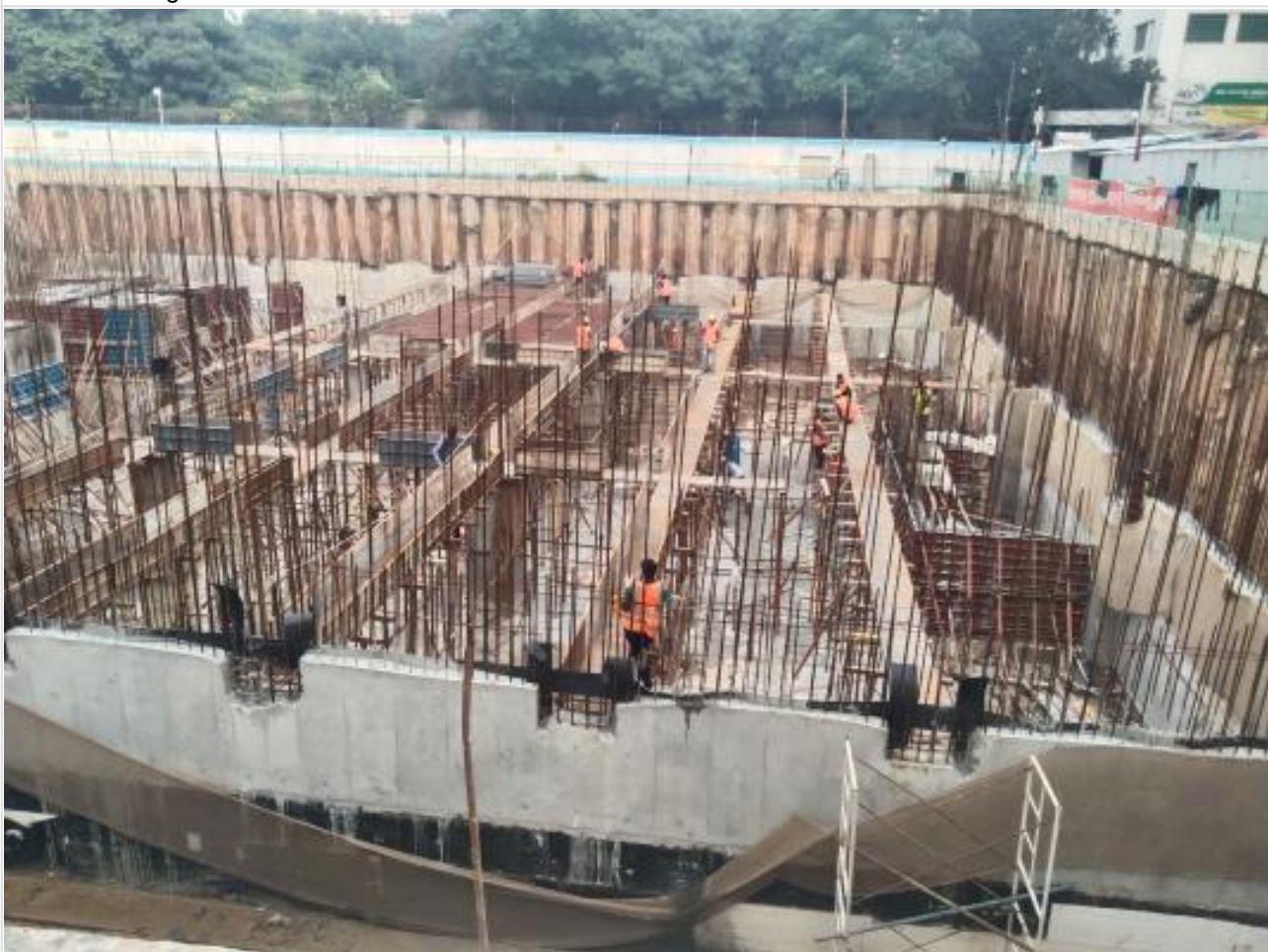
Site picture on 11-12-21
