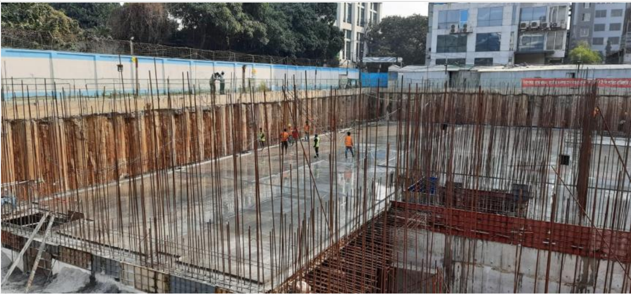
Retaining wall rrbarr work on 20-01-22
