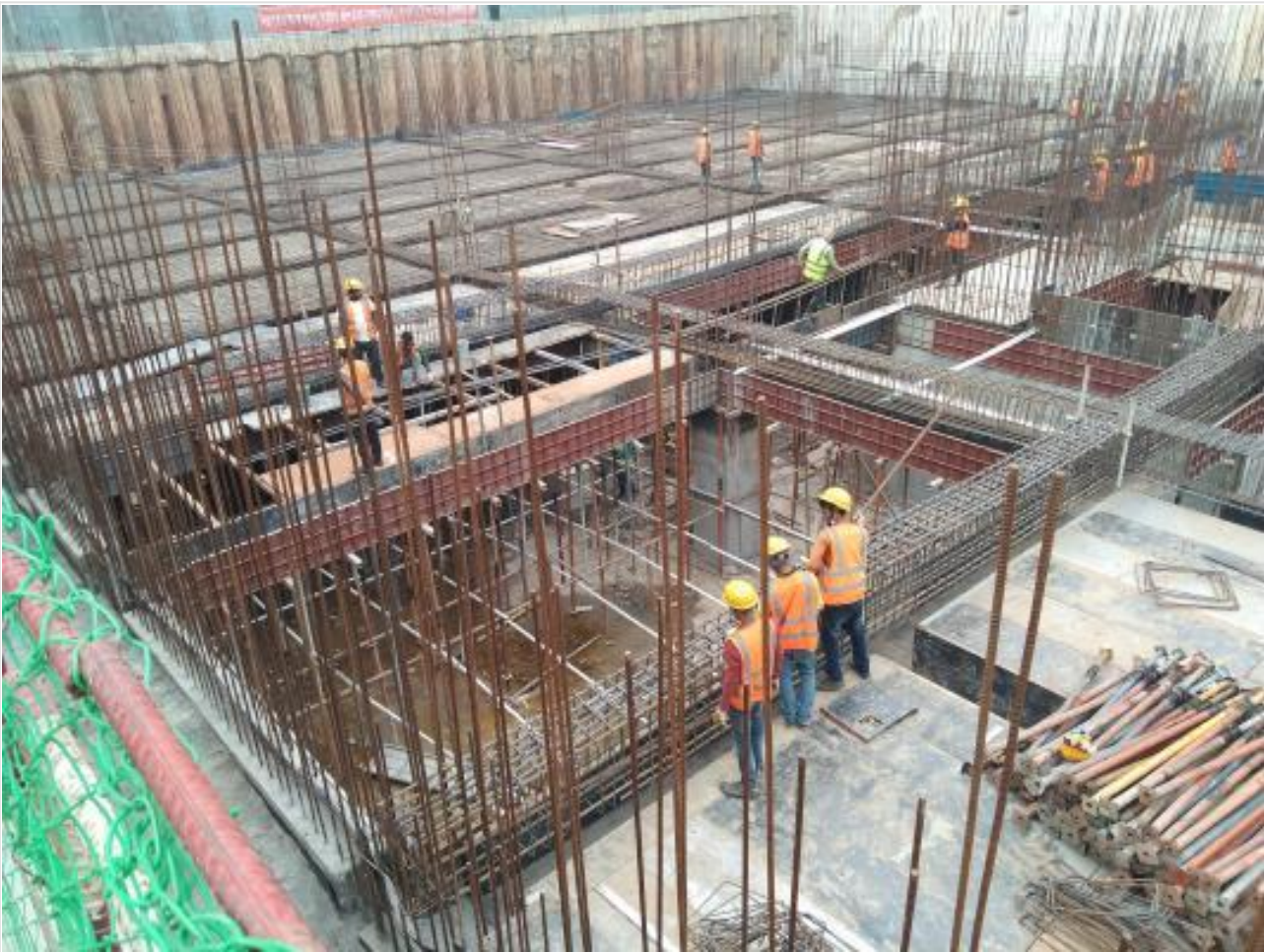
Basement-1-North Slab Re-bar Work on 02-01-22
