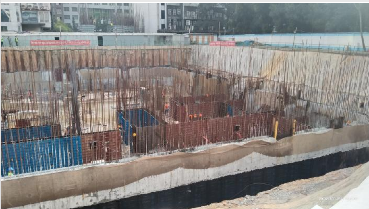
Shear wall and water reserivior shutterin on 24-11-21
