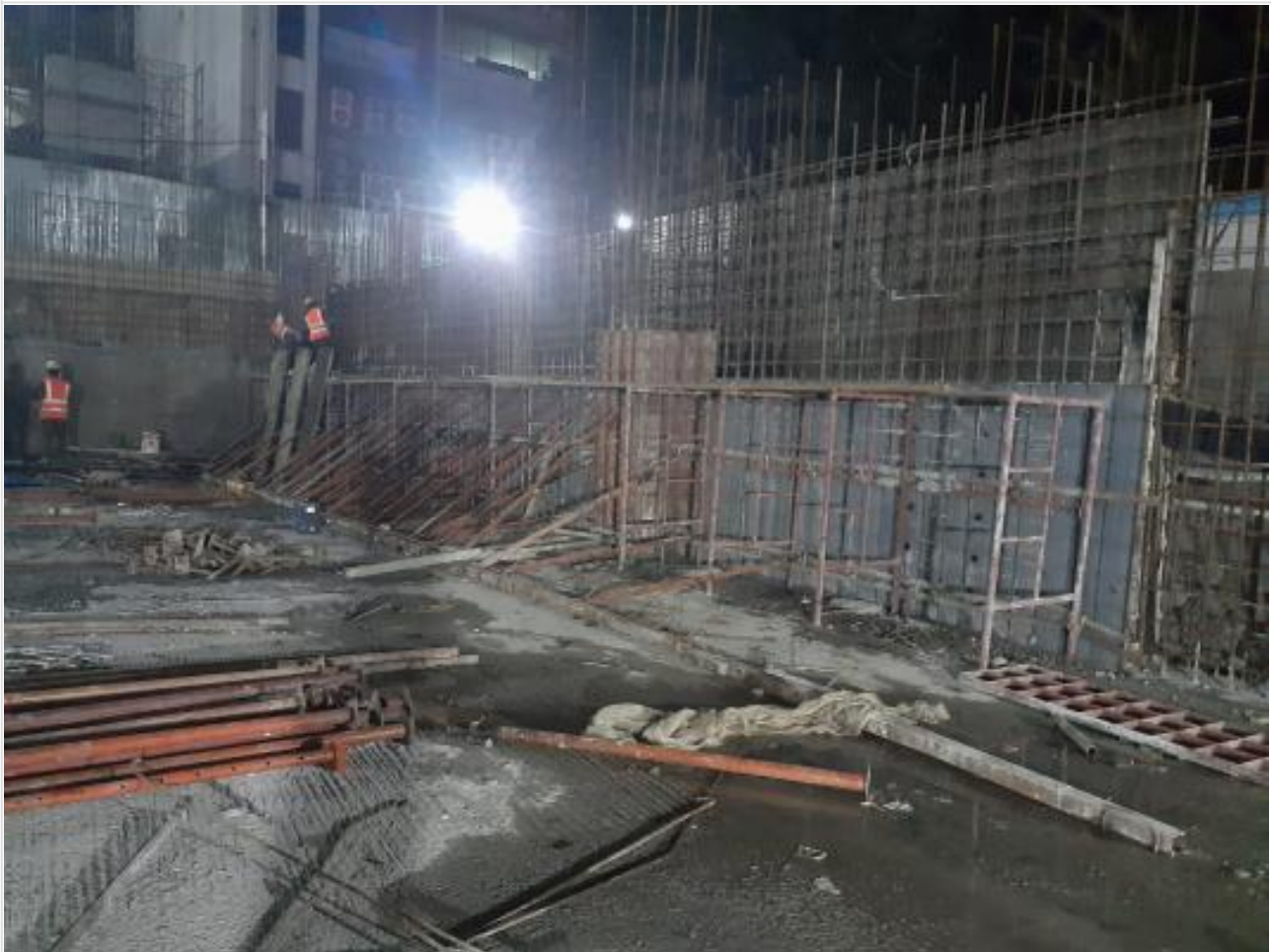
Shuttering work on 18-02-22
