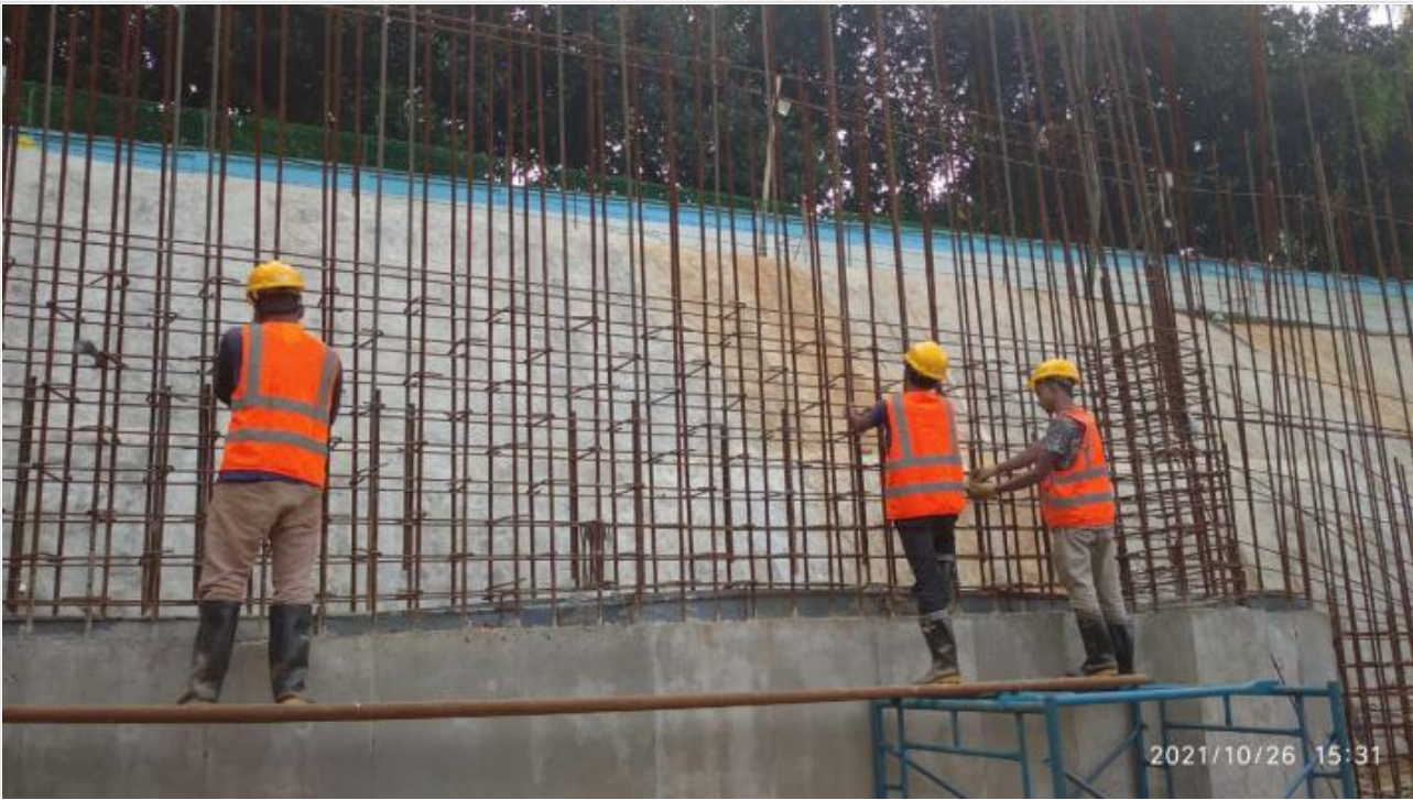
Retaining wall rebar binding on 26-10-21
