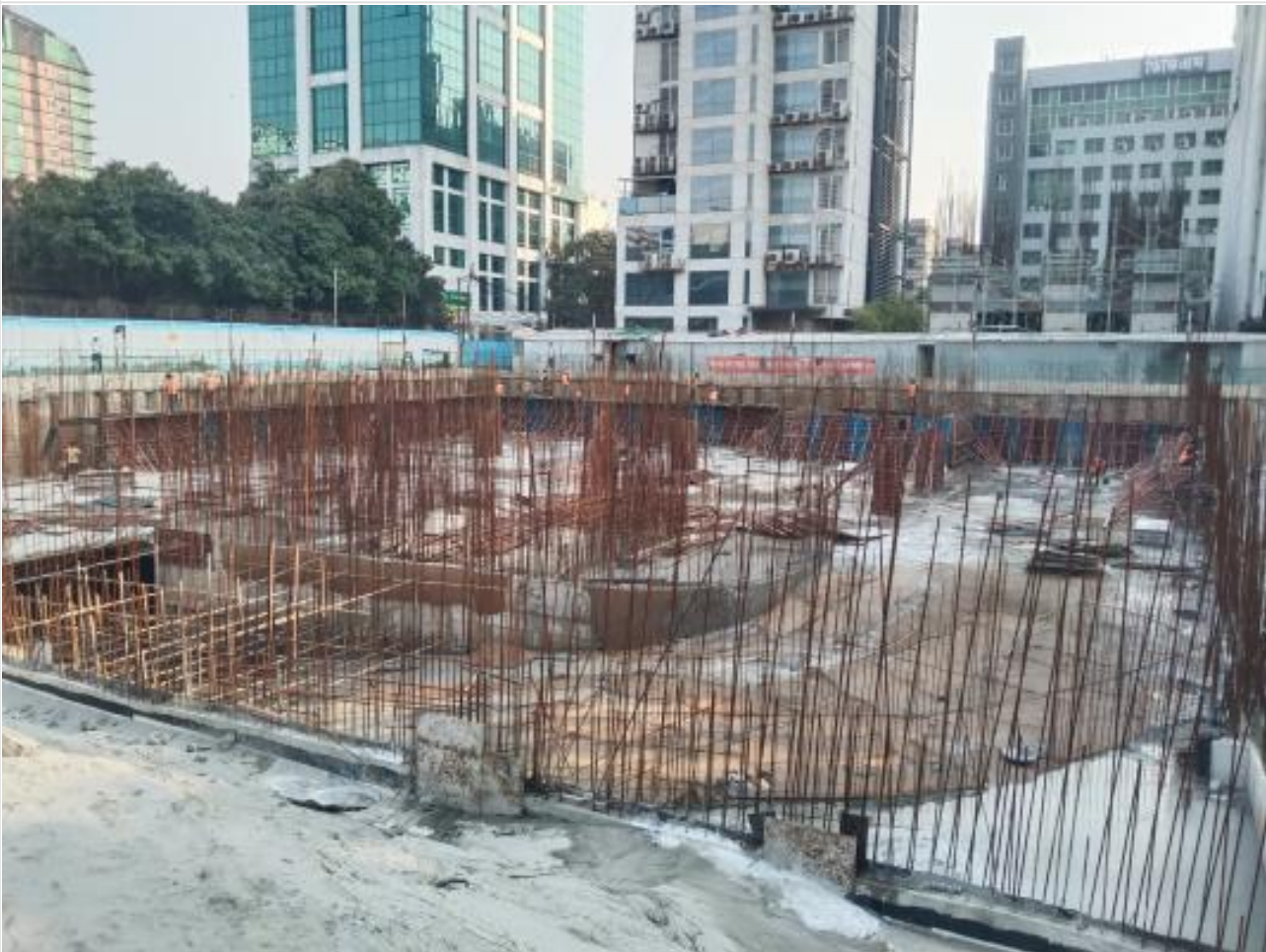
Basement-1-south retaining wall-Re-bar on 16-02-22
