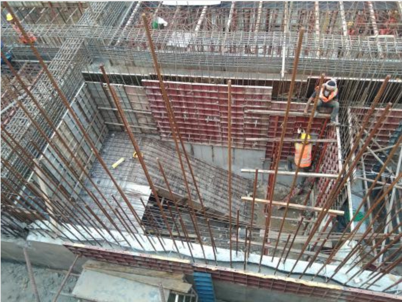
South stair on 19-12-21
