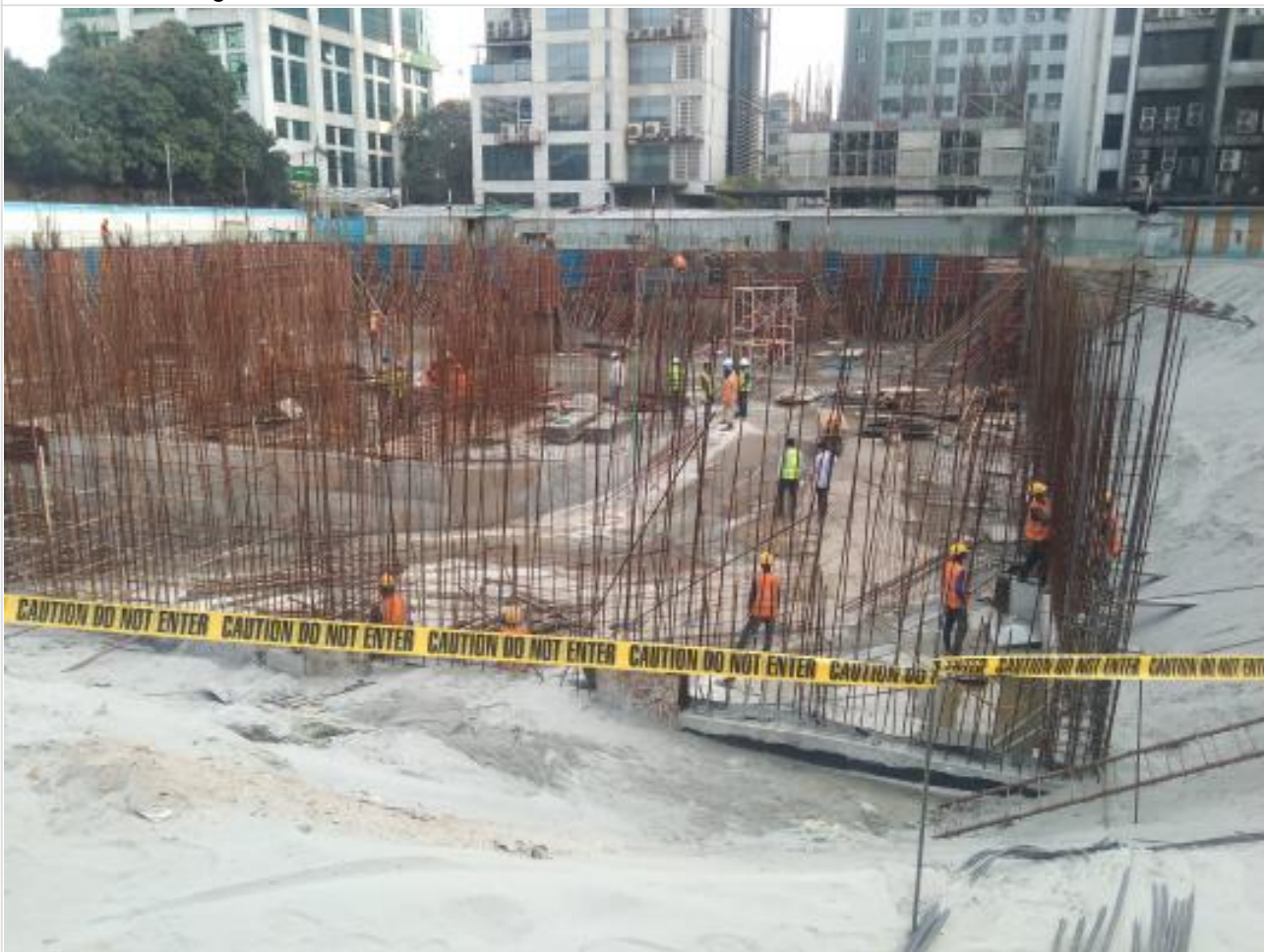
Basement-1-North Retaining wall-1st Lift on 28-02-22
