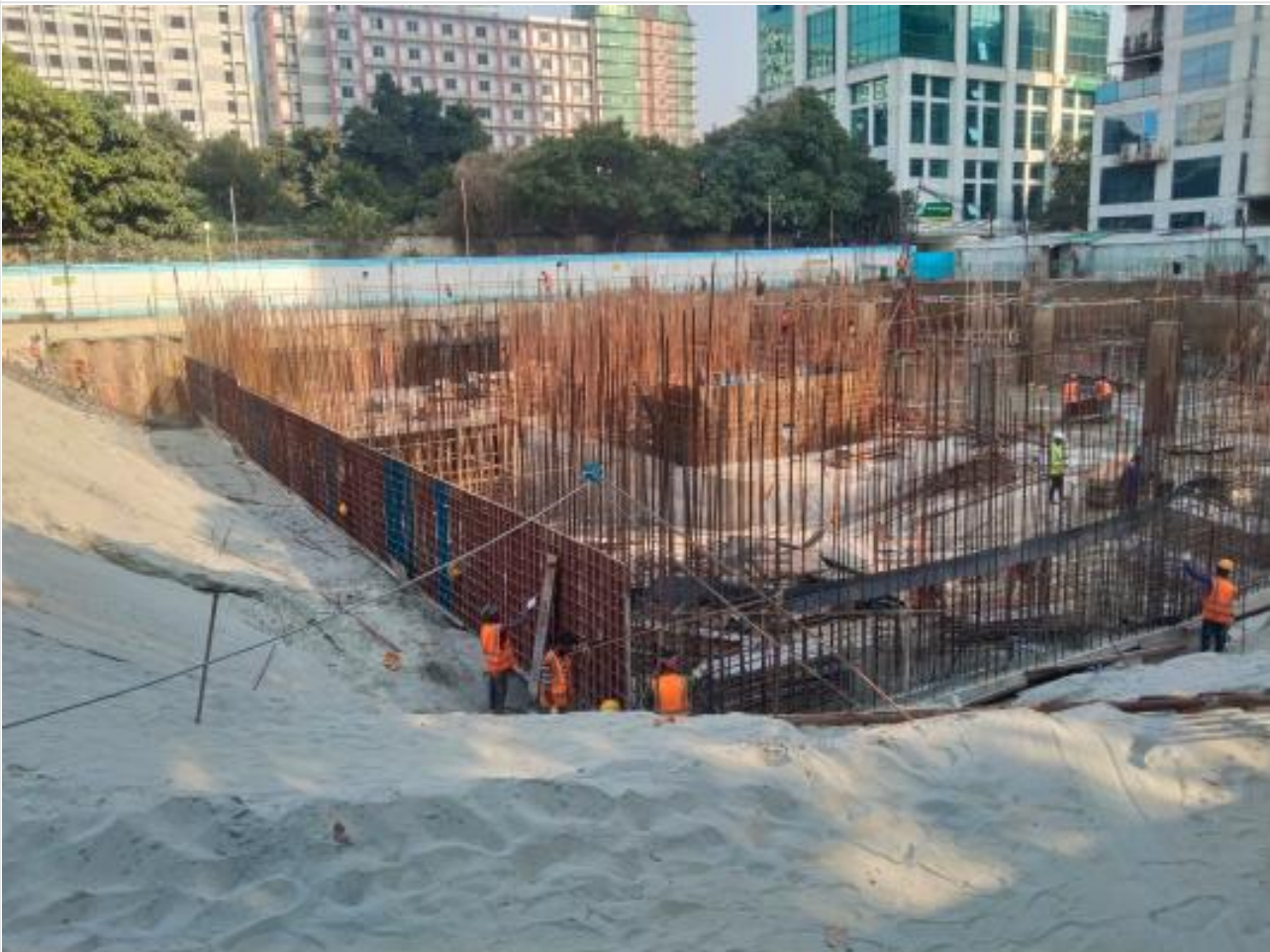
North Retaining wall on 04-03-22
