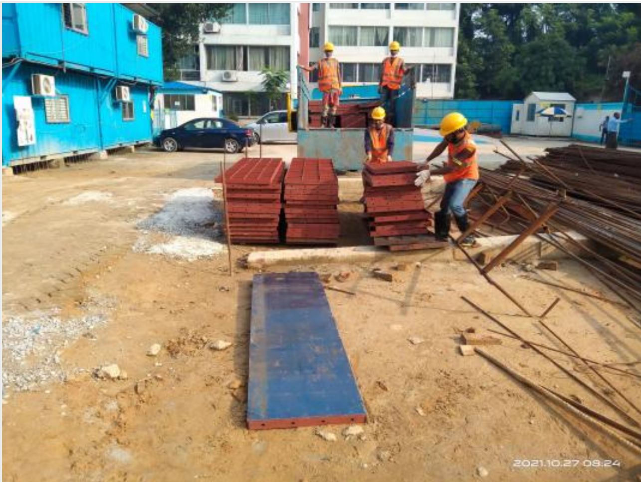
Retaining wall shutter unloading on 27-10-21
