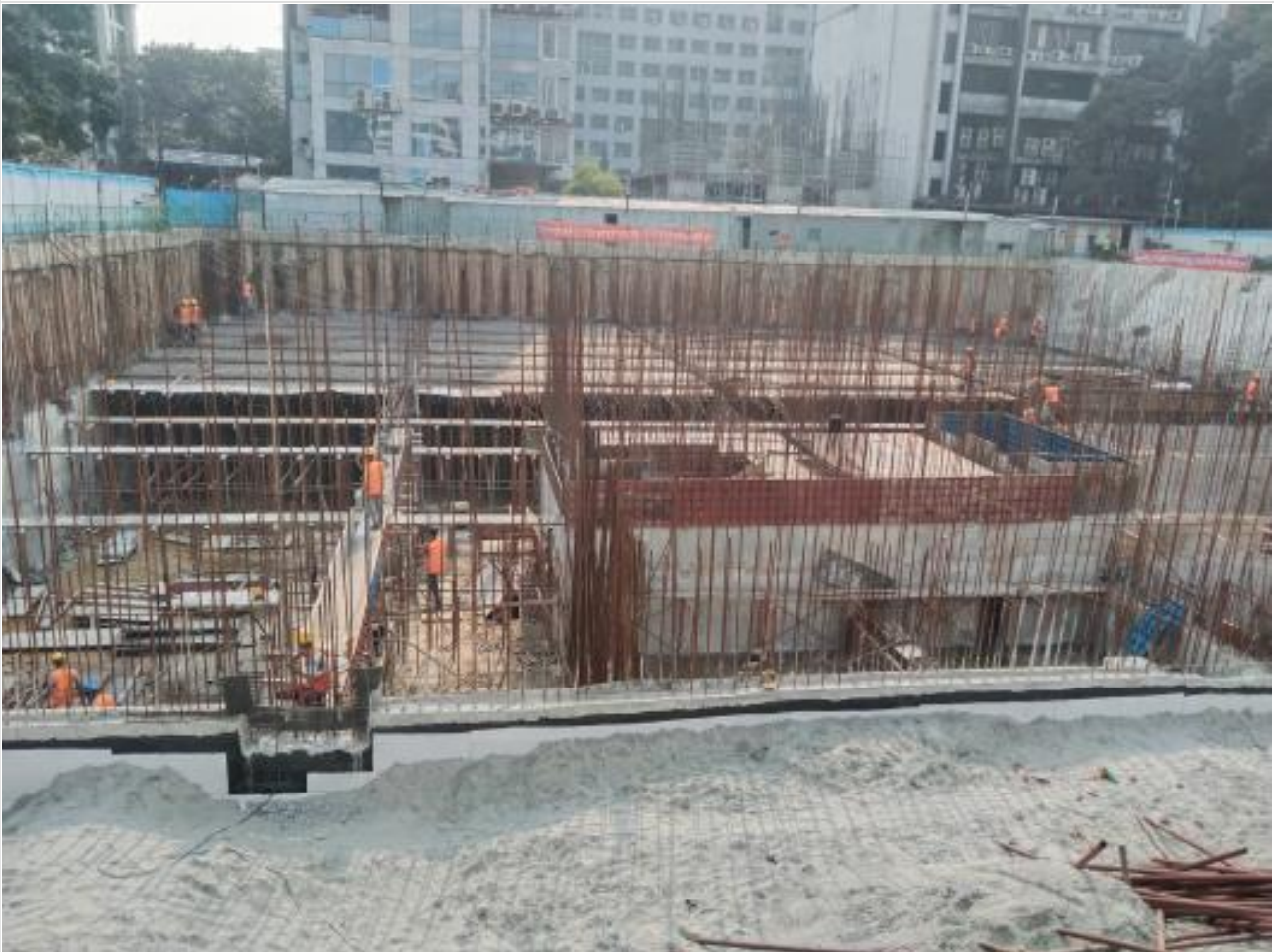
North slab shuttering on 27-12-21
