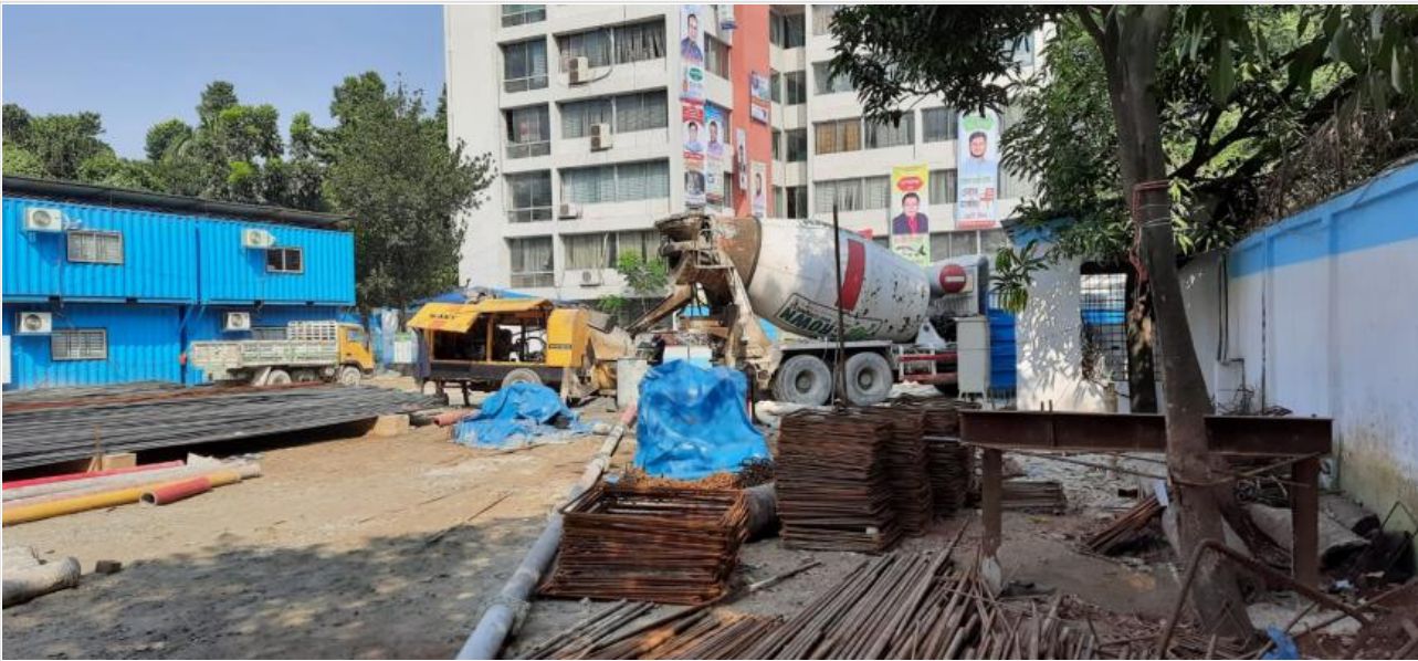
Ready mix concreting with pump on 18-11-21
