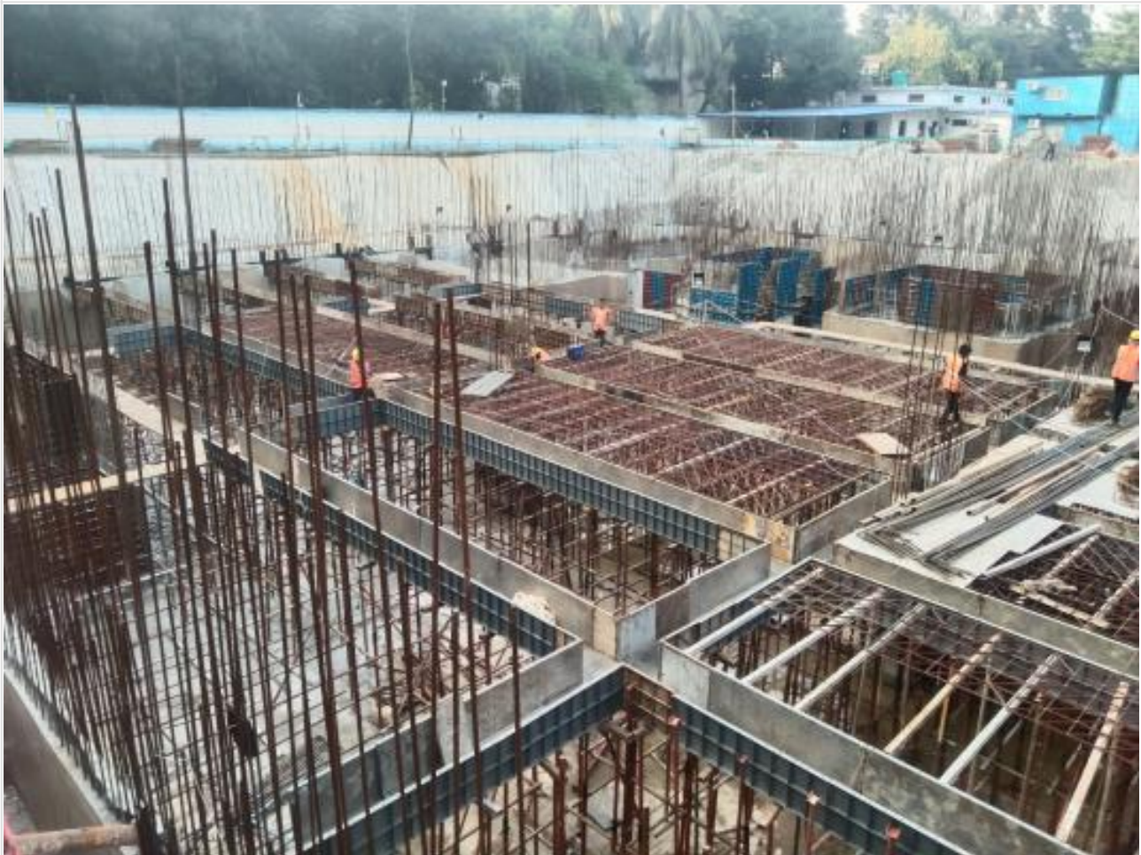
B1 south slab shuttering on 13-12-21
