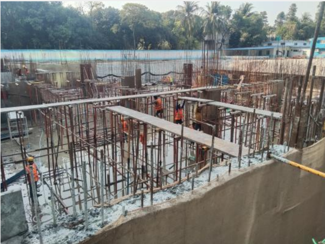
GF slab beam bottom on 04-03-22
