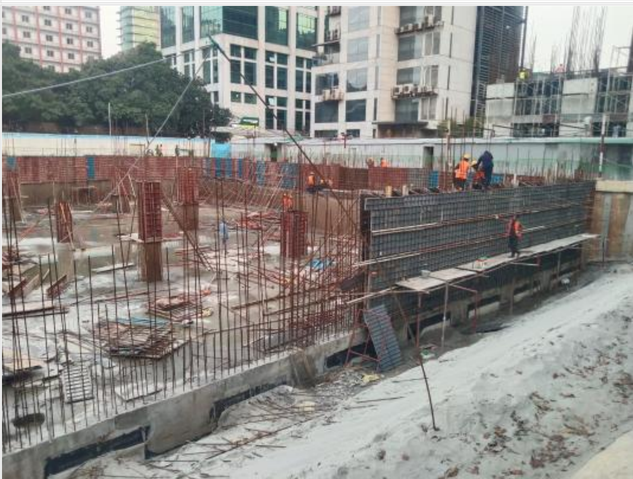
South retaining wall on 22-02-22
