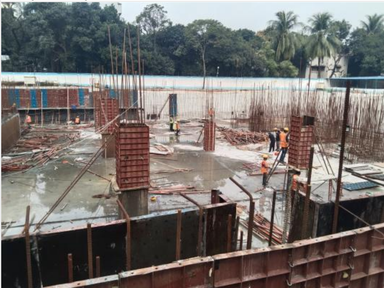
Column shuttering on 20-02-22
