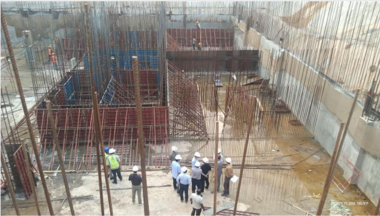
Inspection team on 25-11-21
