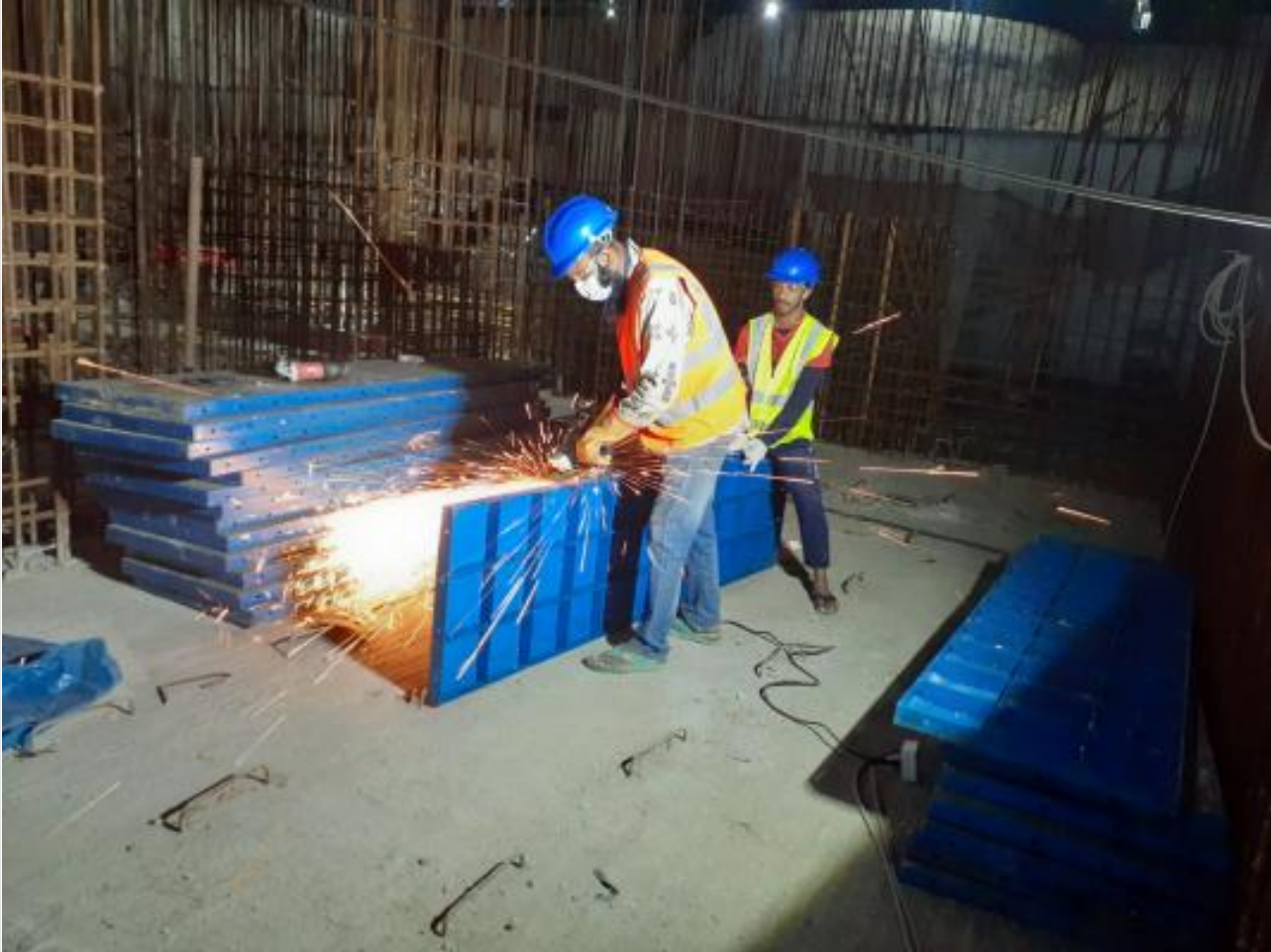
Shear wall shutter carrying to basement on 20-11-21
