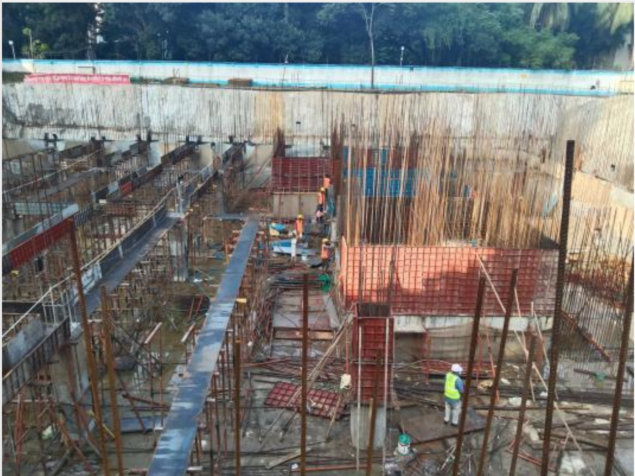
Site picture on 08-12-21
