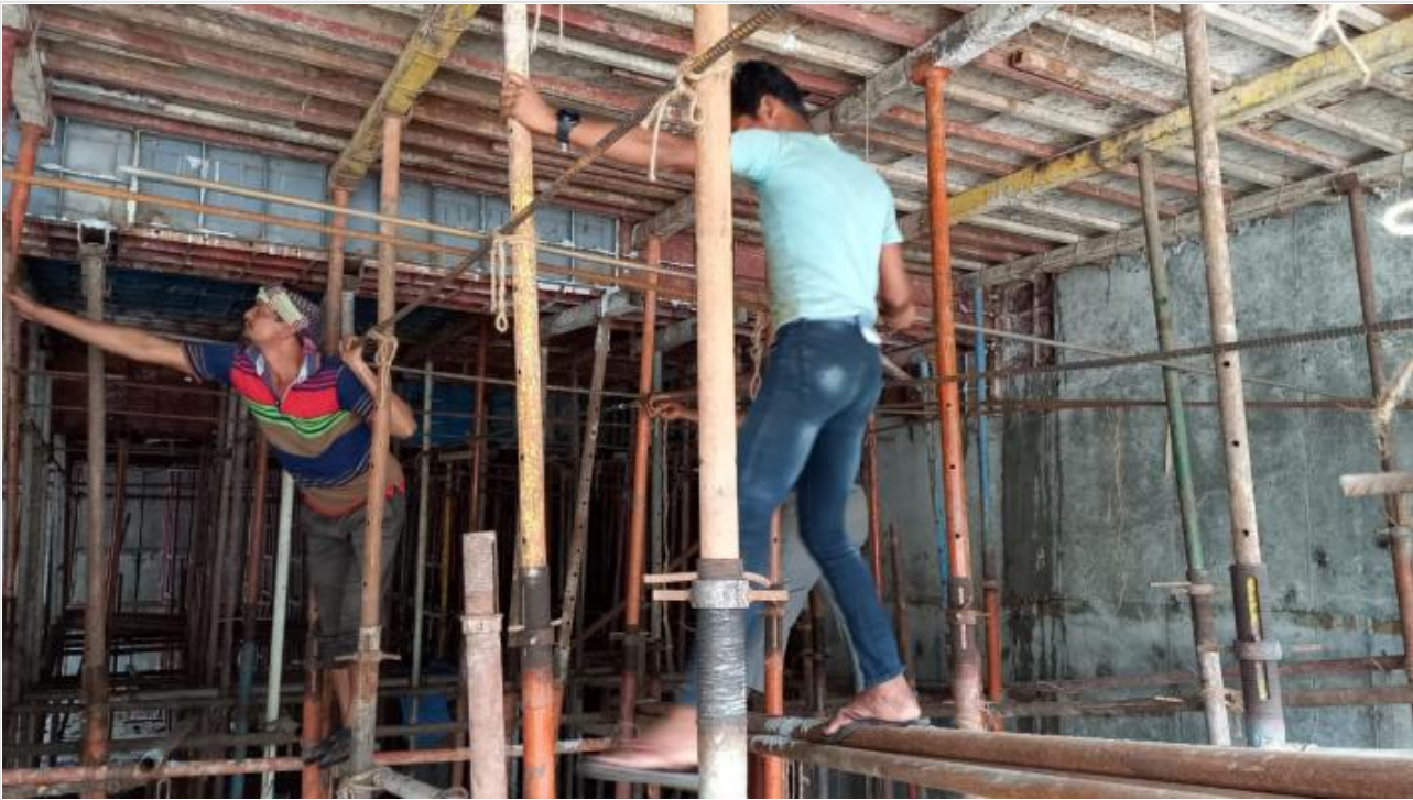
Bracing Remove on 09-05-22
