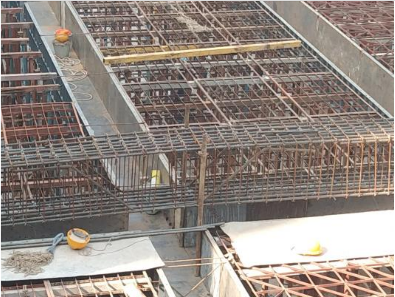
South slab shuttering and rod binding on 15-12-21
