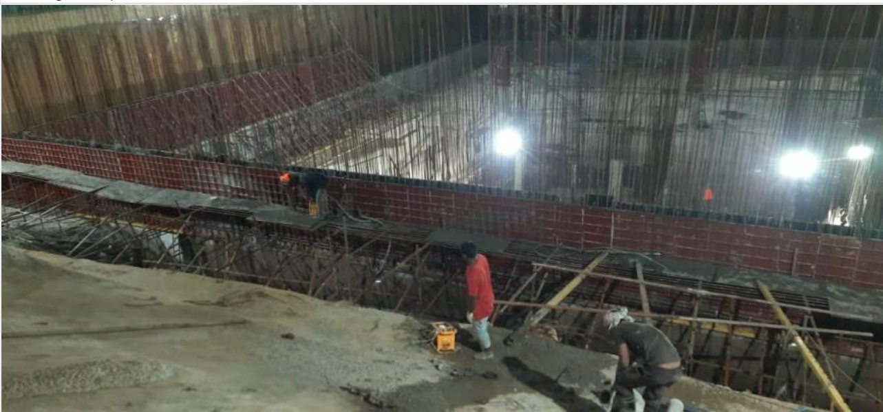
Casting finishing picture on 12-11-21
