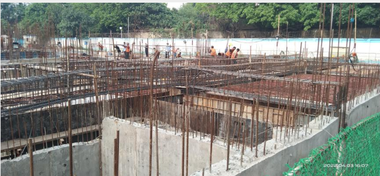
GF slab work progress on 03-04-22
