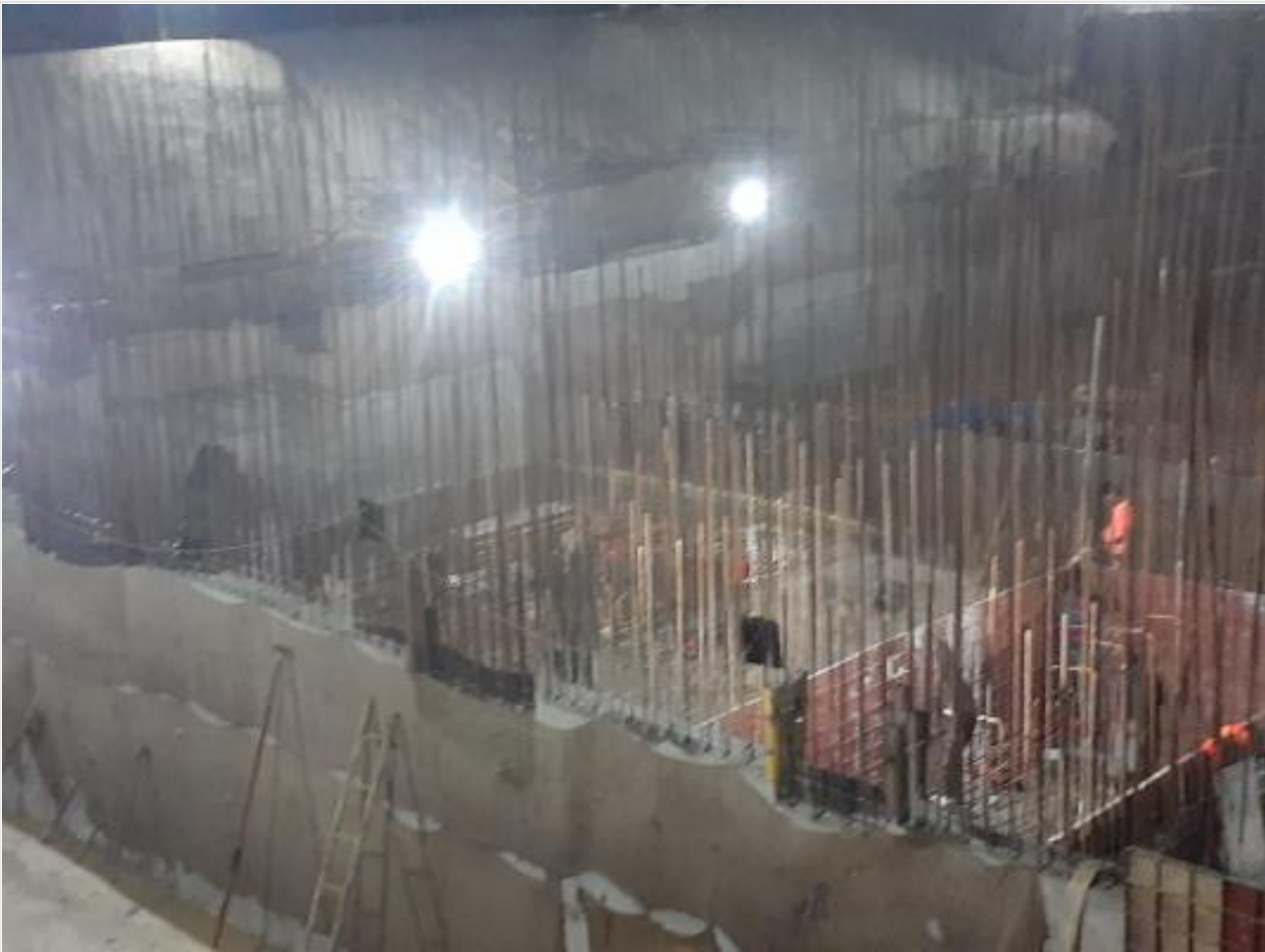
Night work on 21-11-21
