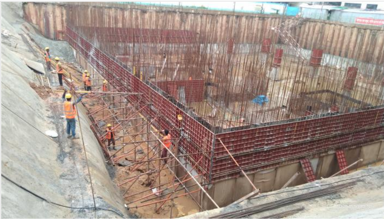
Site picture on 14-11-21
