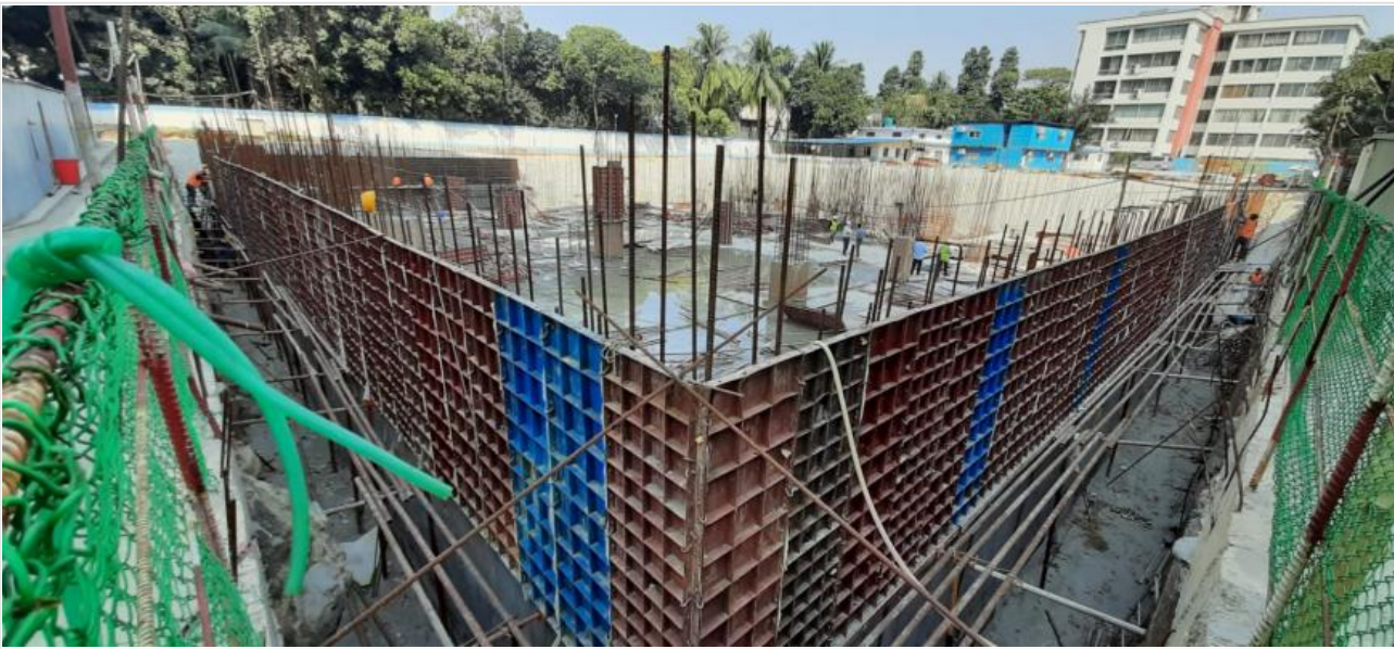
South 2nd lift retaining wall on 18-02-22
