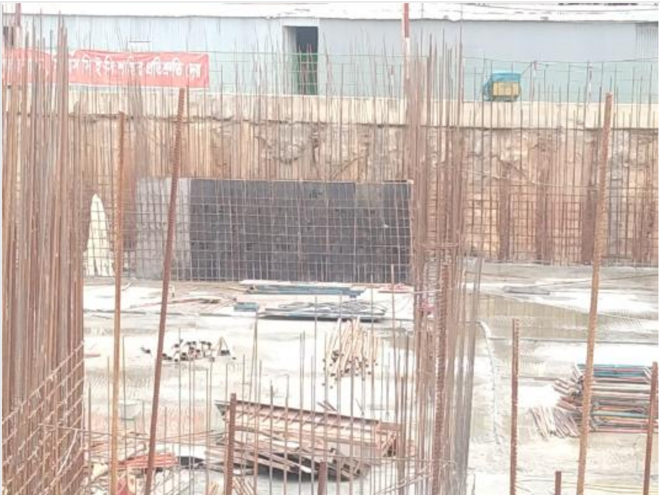
South stair shutter on 03-02-22
