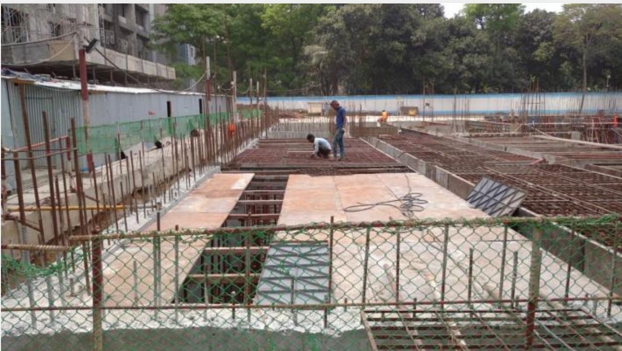
Slab shuttering on 23-03-22
