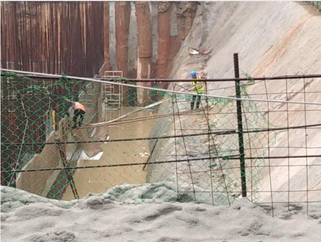
Prepared for water discharge on 06-12-21
