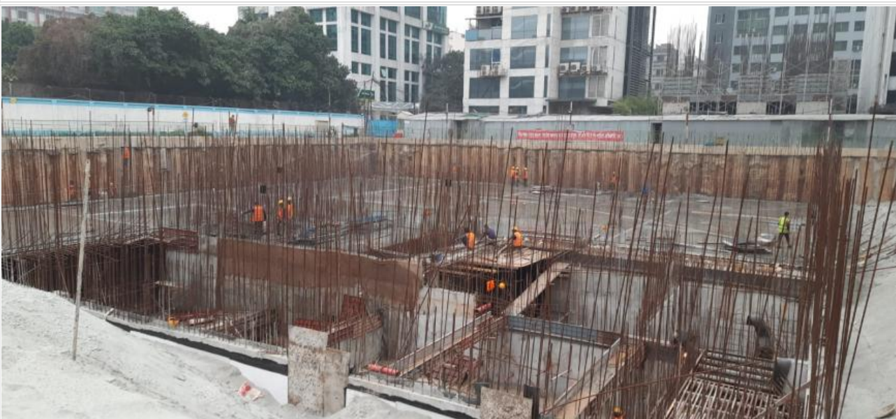
Rebar work on 24-01-22
