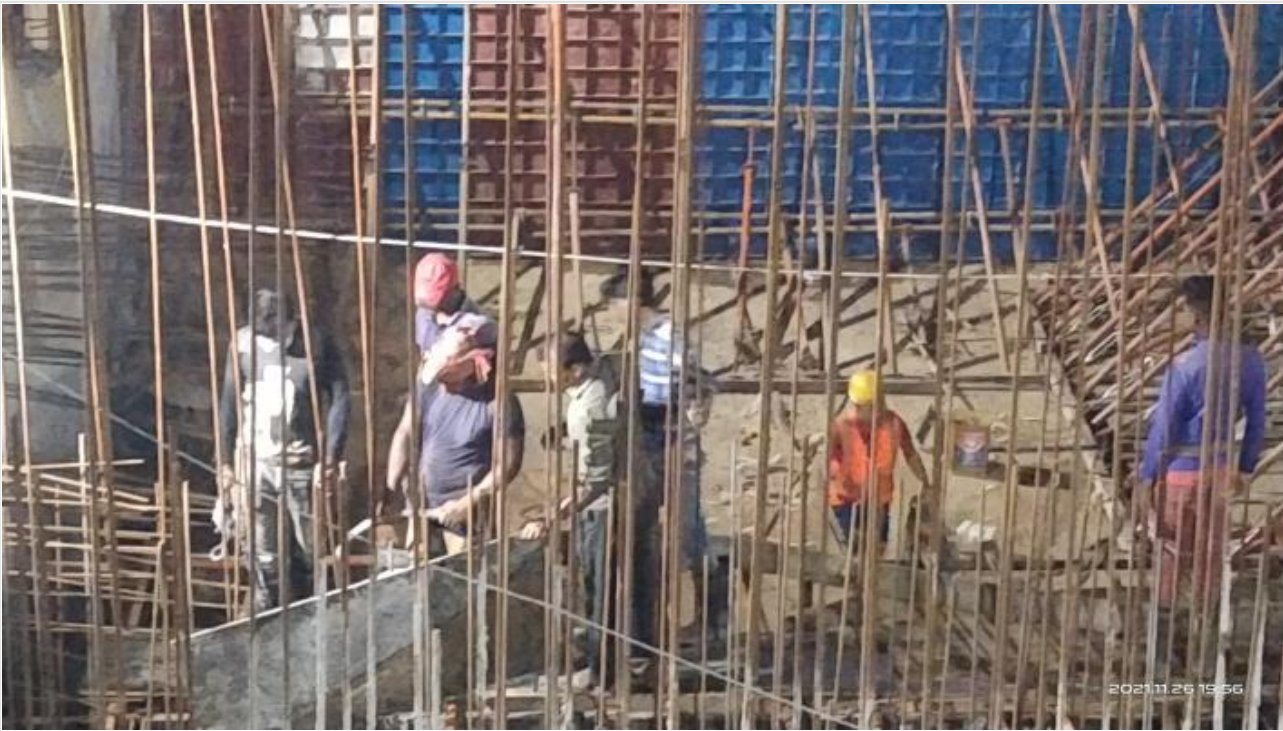
Concreting work on 26-11-21
