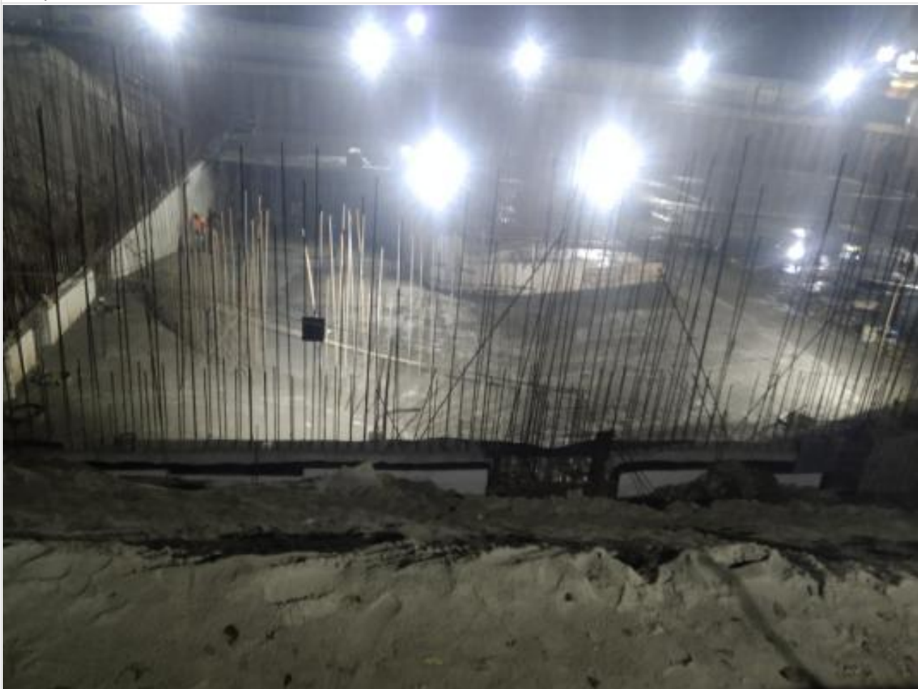
Ramp concreting on 30-01-22
