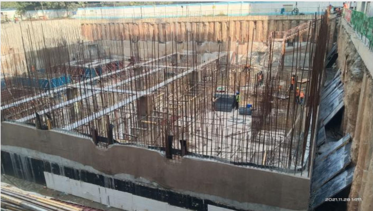
B1 Slab beam bottom shutter on 28-11-21
