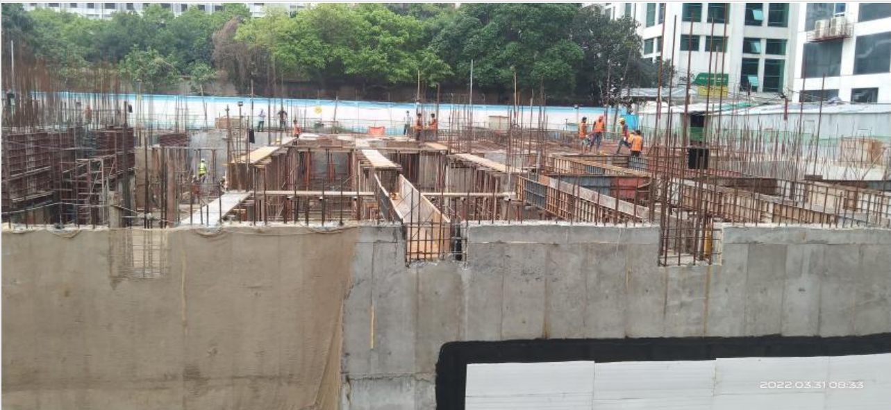
Ground Floor Beam Rebar binding on 31-03-22
