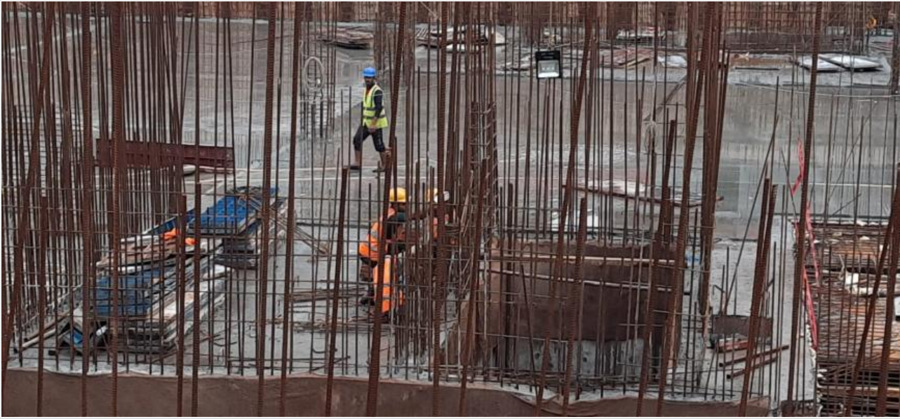
Ramp shuttering on 24-01-22
