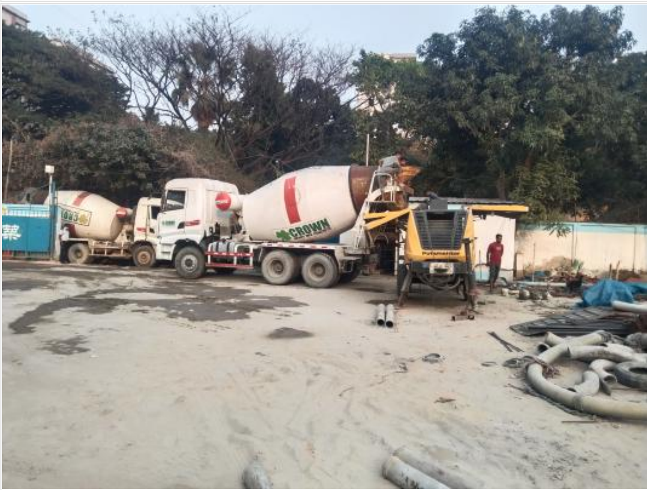
Ready-mix Concrete Truck and Pump on 26-02-22
