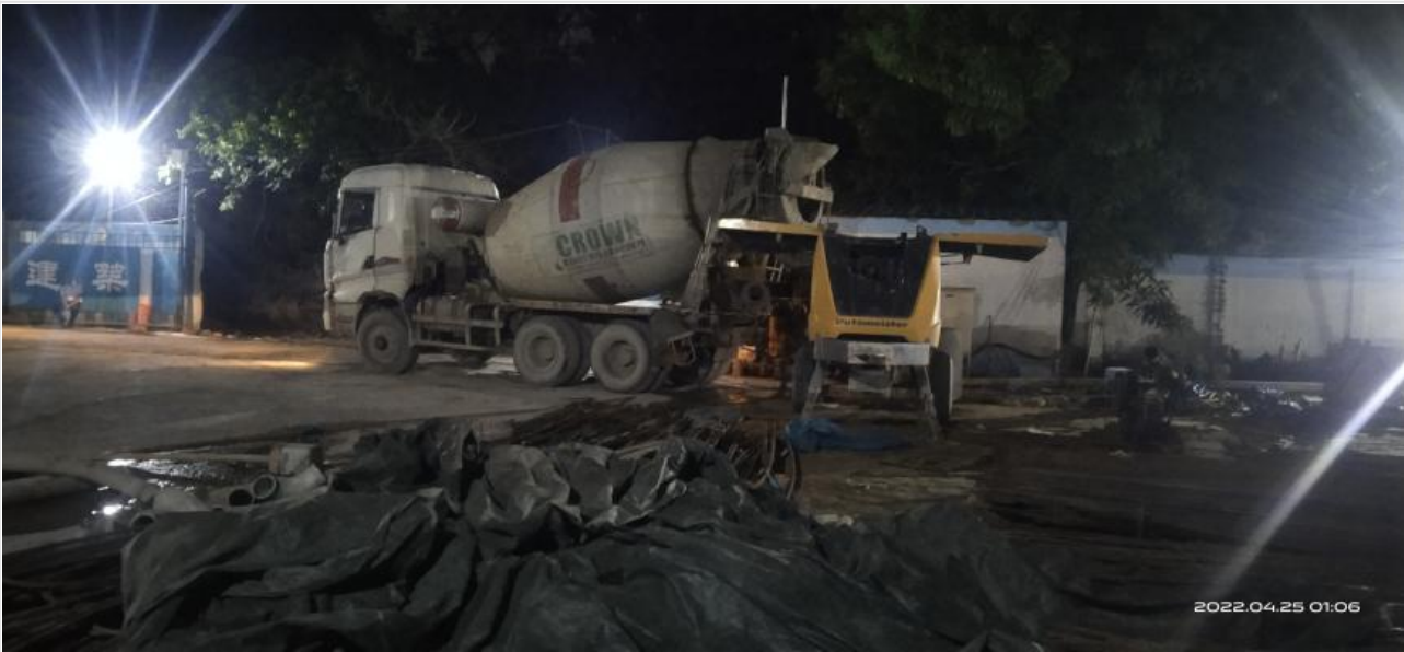
Ready mix Concrete Truck on 24-04-22
