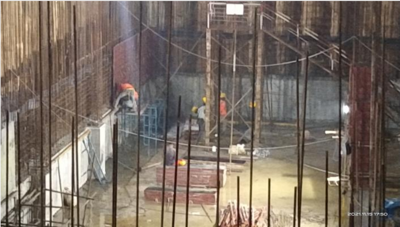
Shuttering at night on 15-11-21
