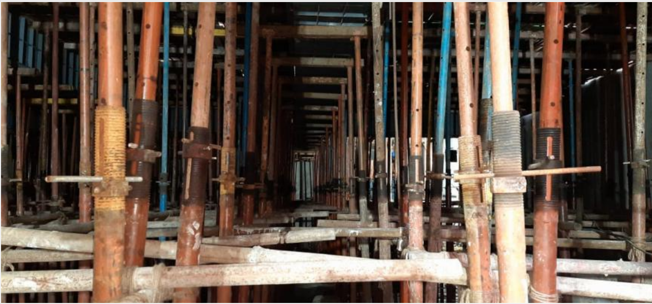
Slab levelling work on 12-01-22
