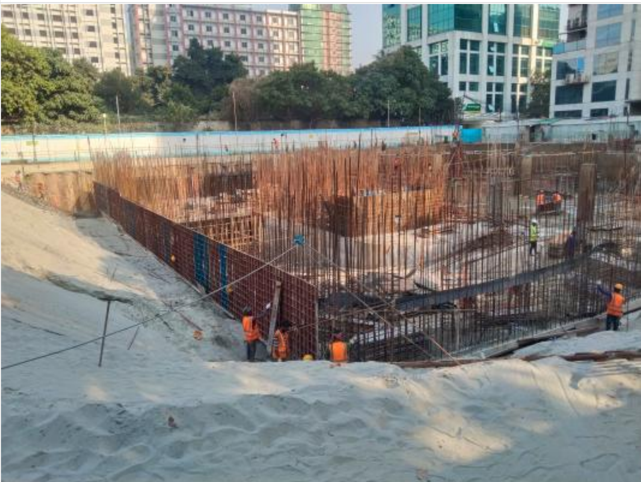
North Retaining wall on 04-03-22
