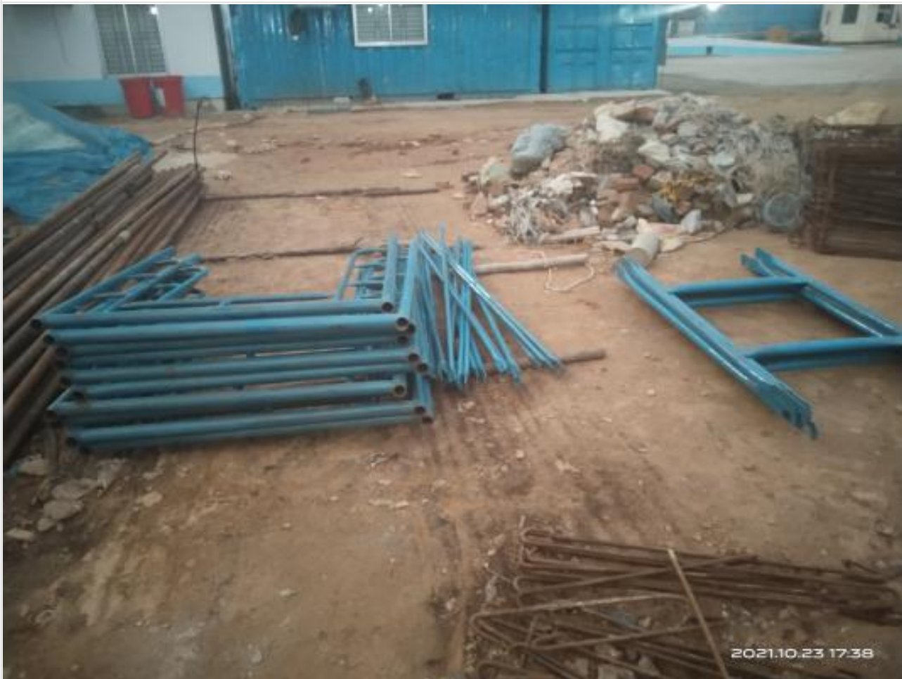
Scaffolding Materials received at site on 23-10-21
