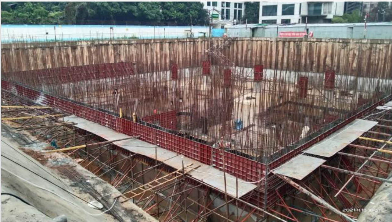
Site picture on 13-11-21
