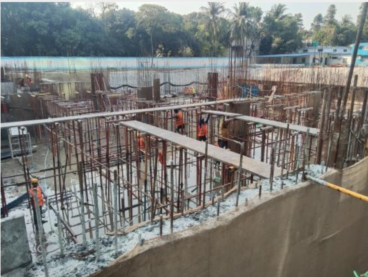
GF slab beam bottom on 04-03-22
