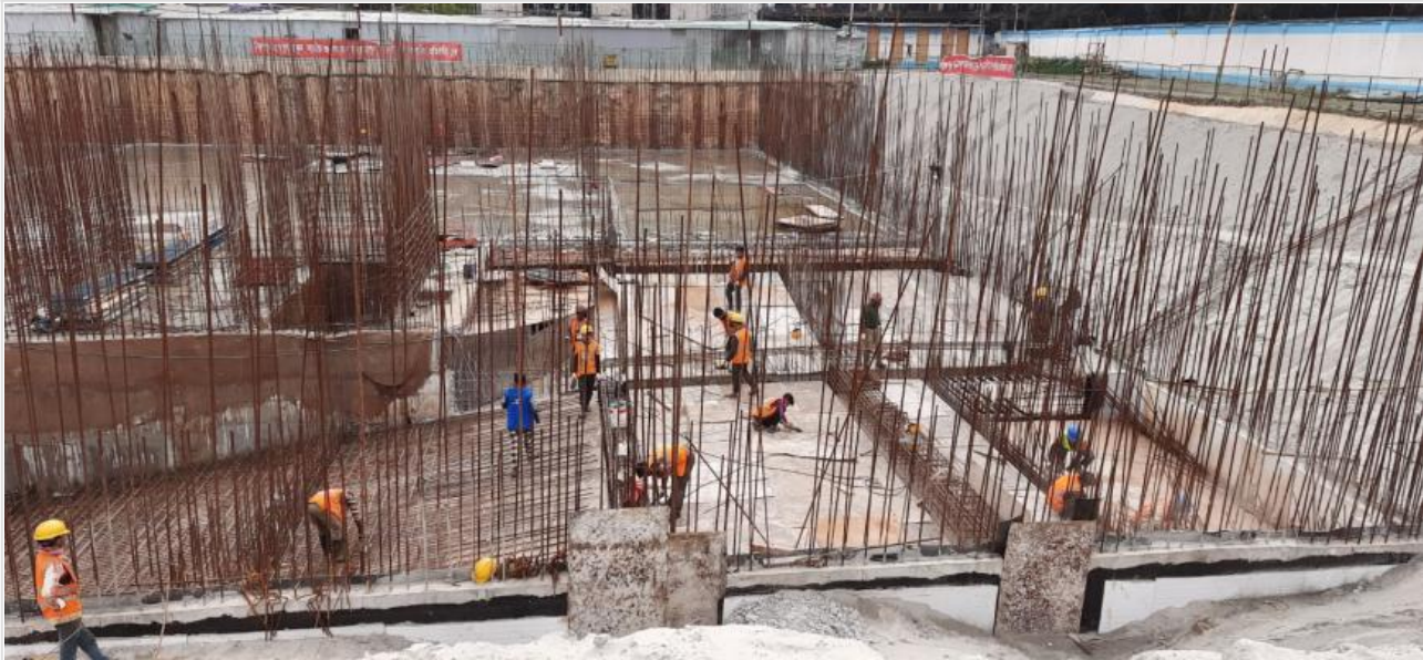
Ramp work on 28-01-22
