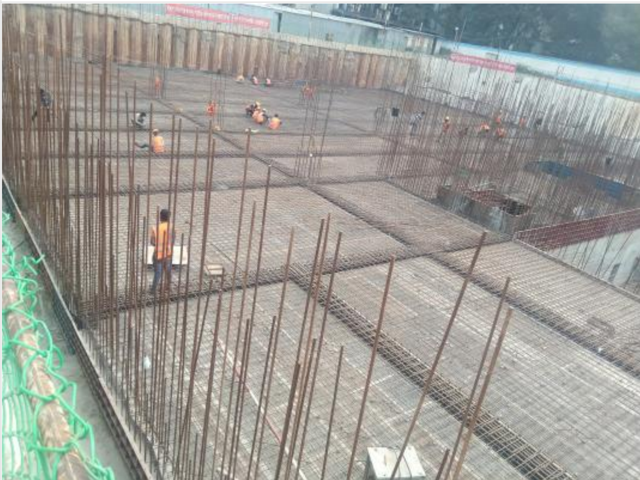
North south slab on 11-01-22
