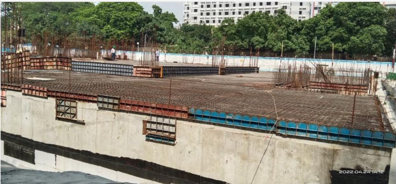
Slab inspection on 23-04-22
