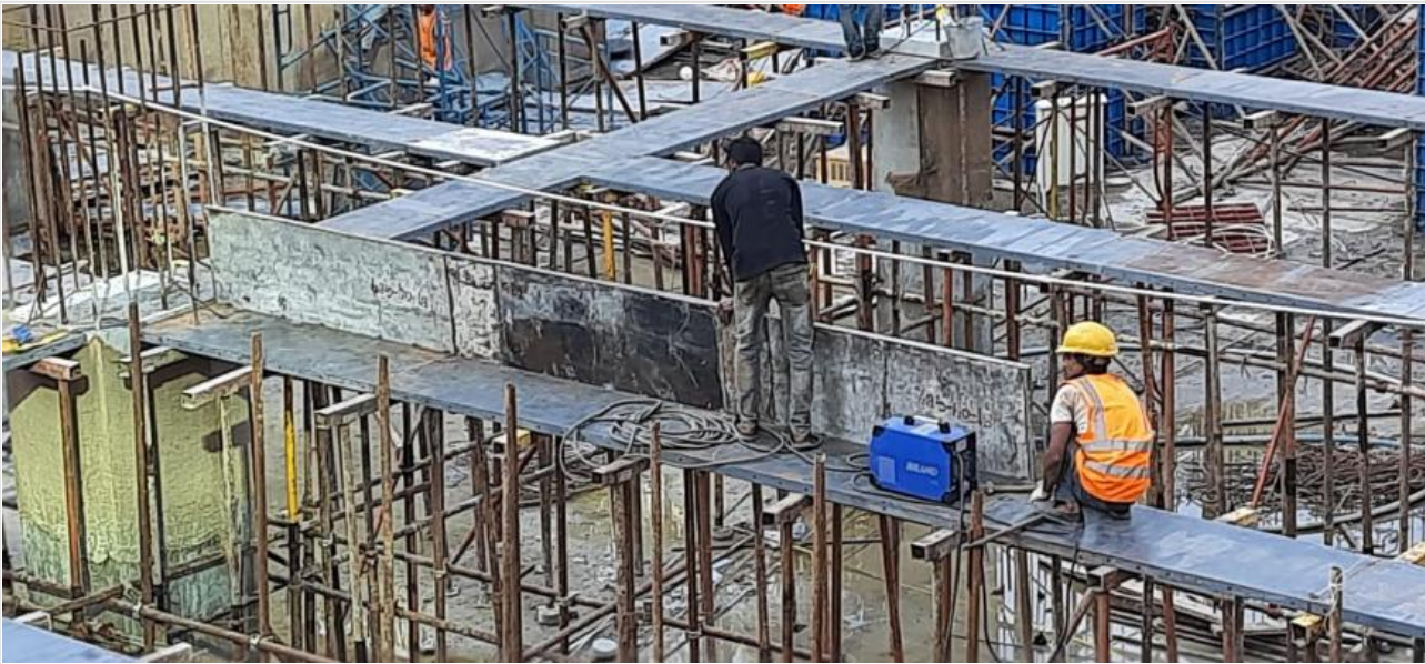
Slab shuttering on 30-11-21
