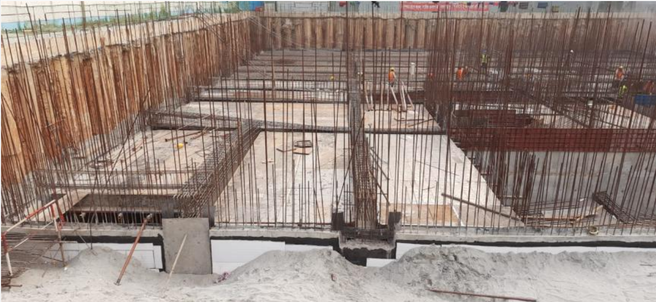
North slab work on 04-01-22
