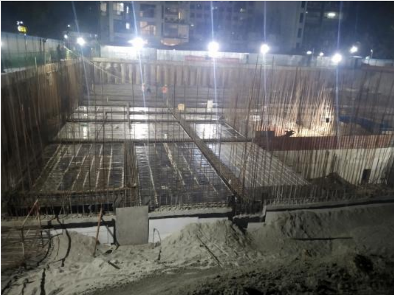
Basement-1-Slab shuttering on 05-01-22
