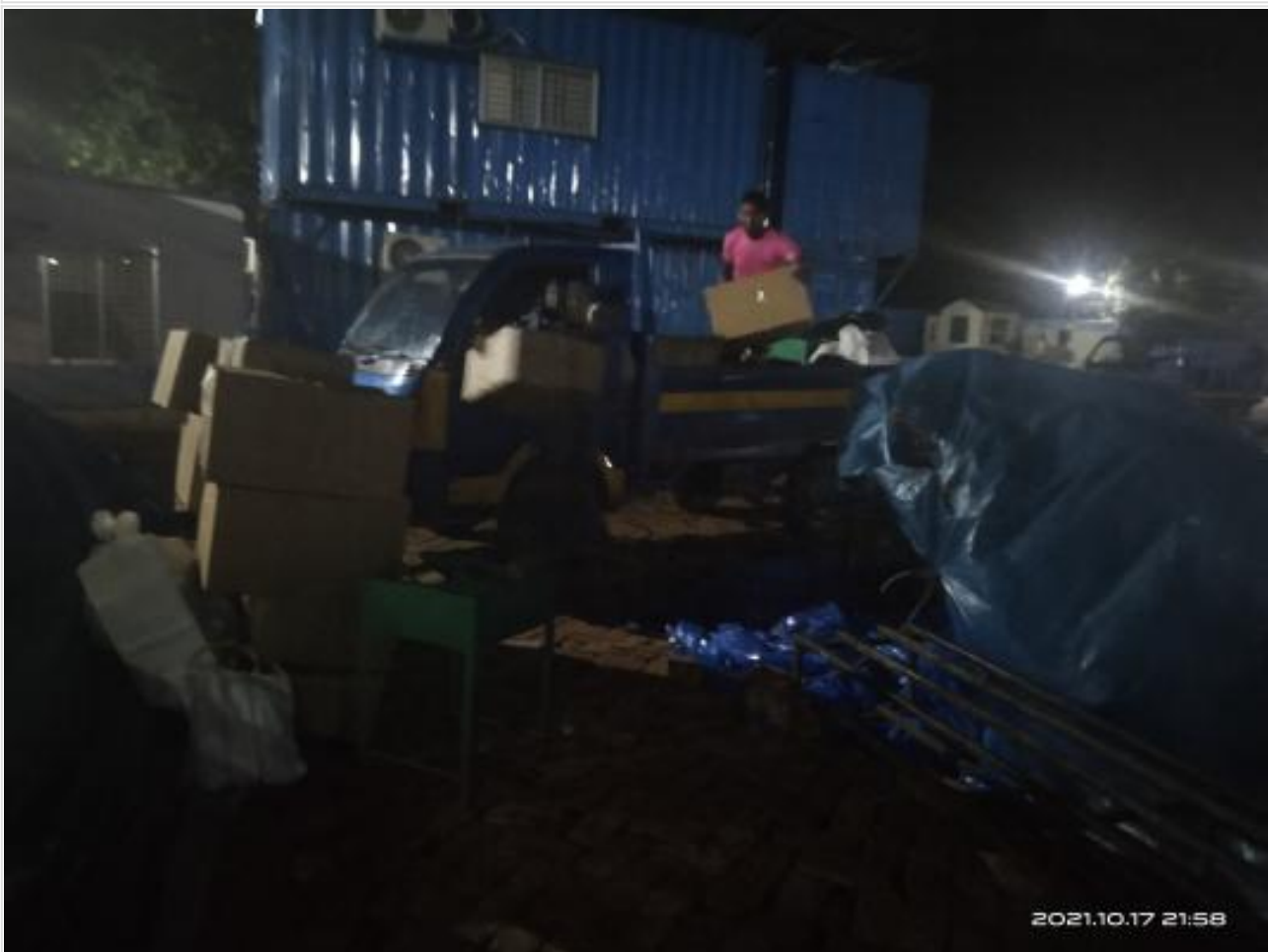
Materials mobilization (Received) on 17-10-21
