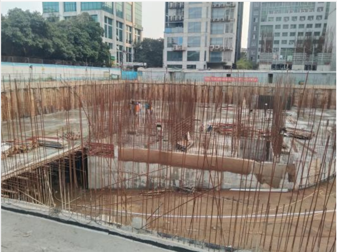
Overall site on 03-02-22
