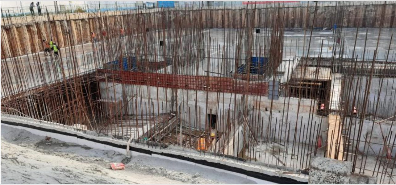
Ramp shuttering work on 20-01-22
