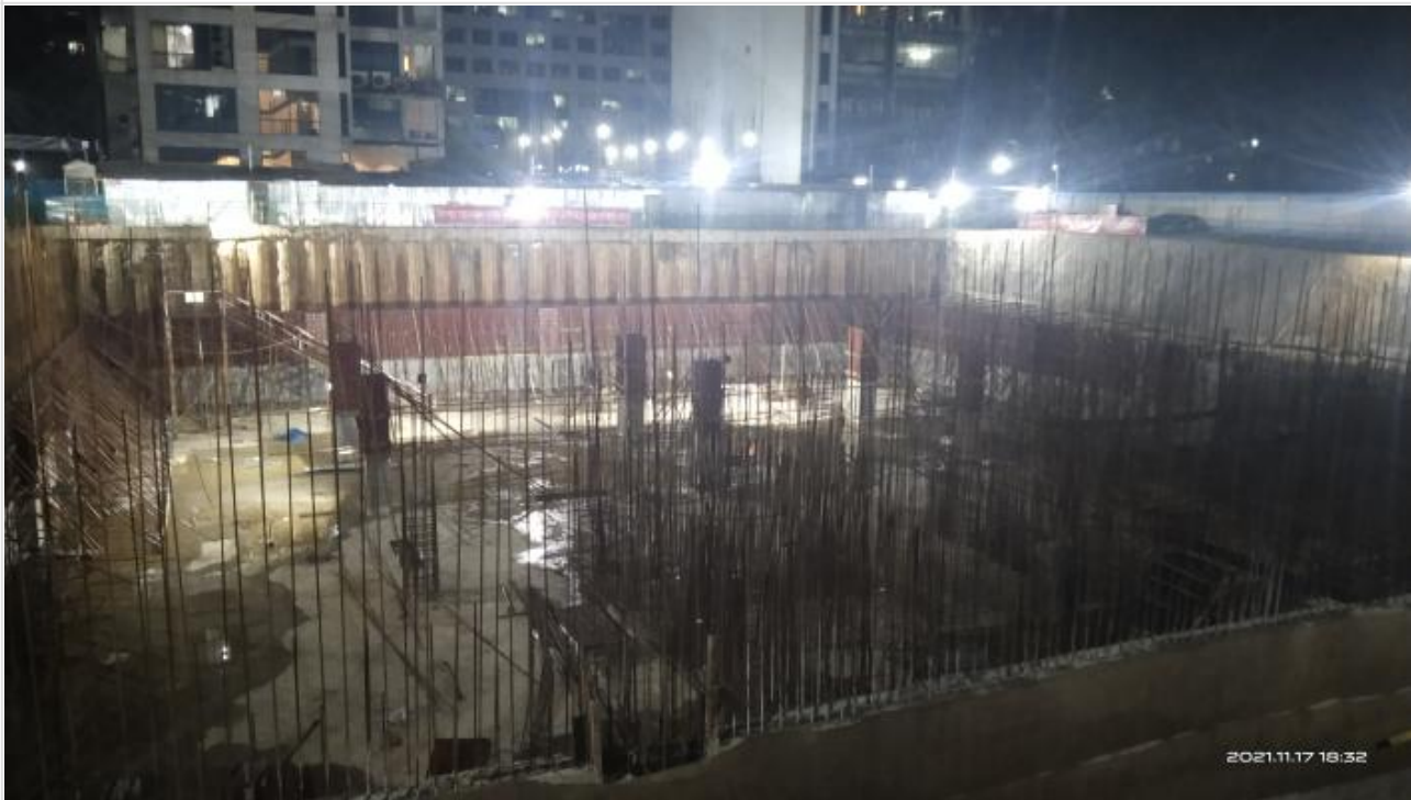
Retaining wall work progress on 17-11-21
