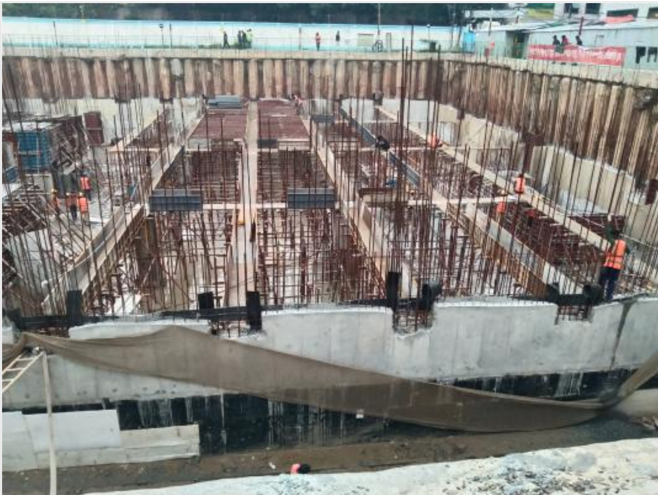
Slab shuttering work on 11-12-21
