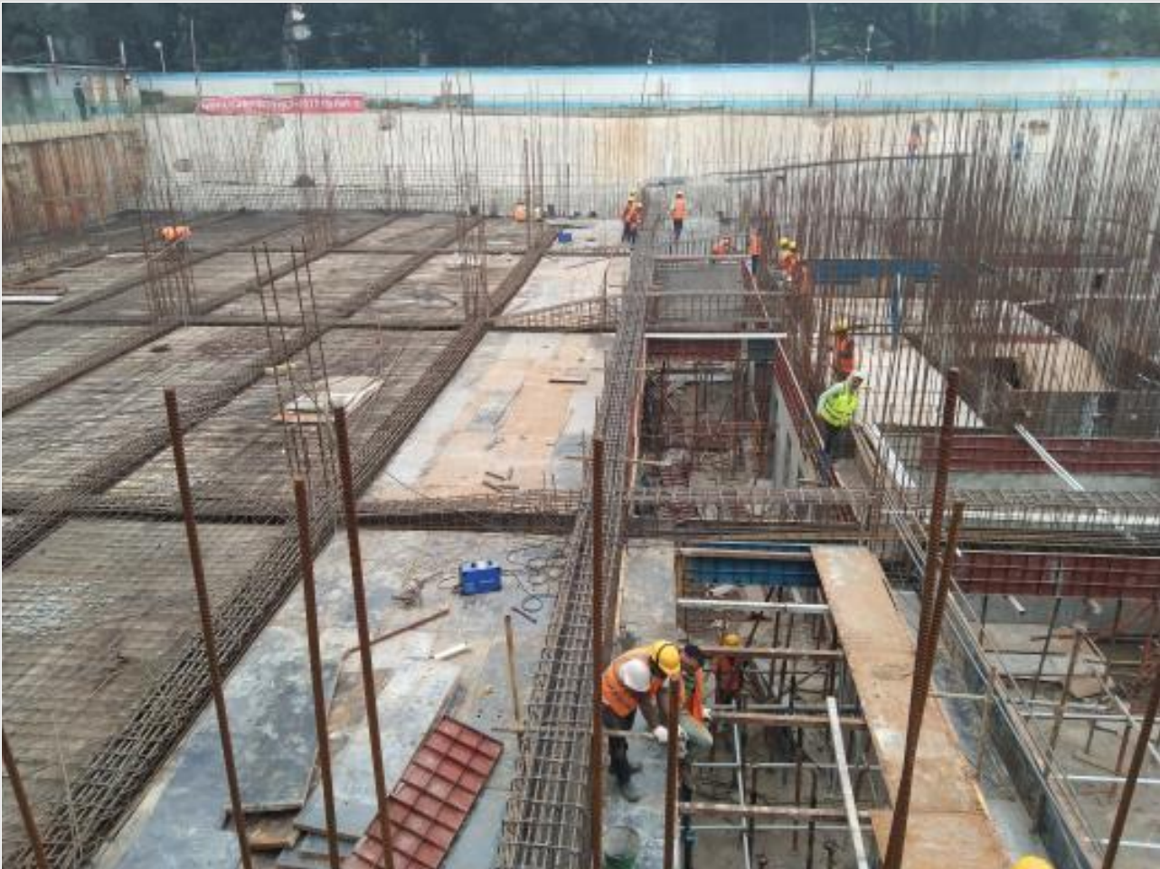
Basement-1-North Slab Re-bar Work on 02-01-22
