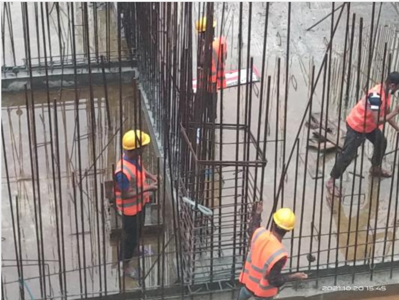
Column ring rod binding on 20-10-21
