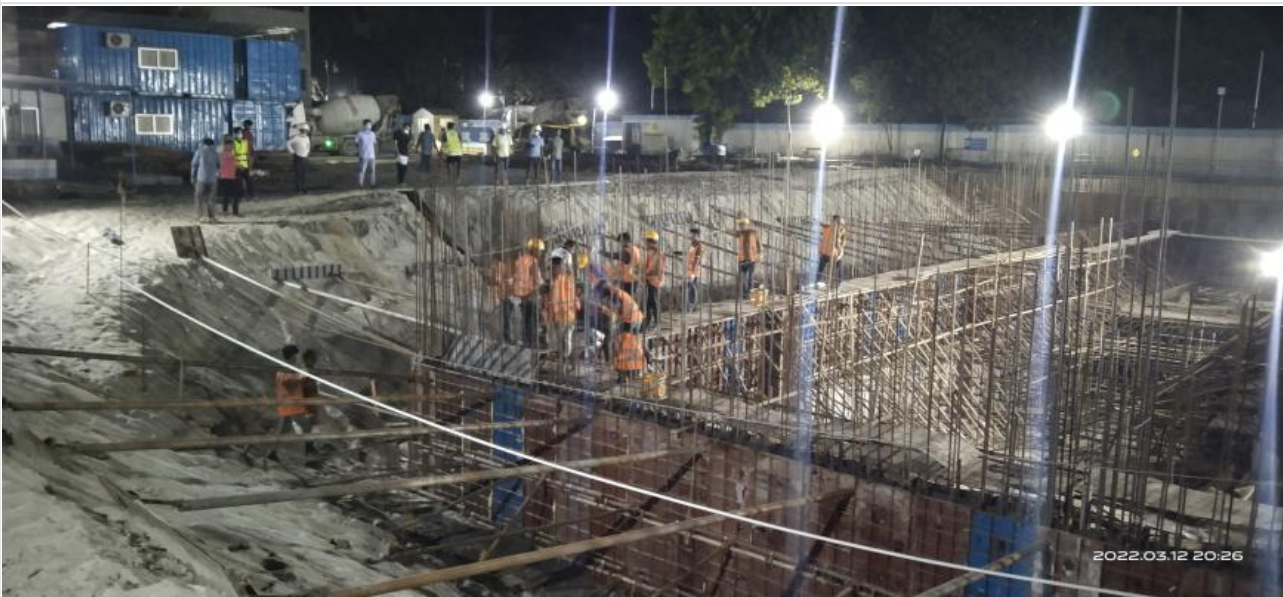
Ready mix concreting on 13-03-22
