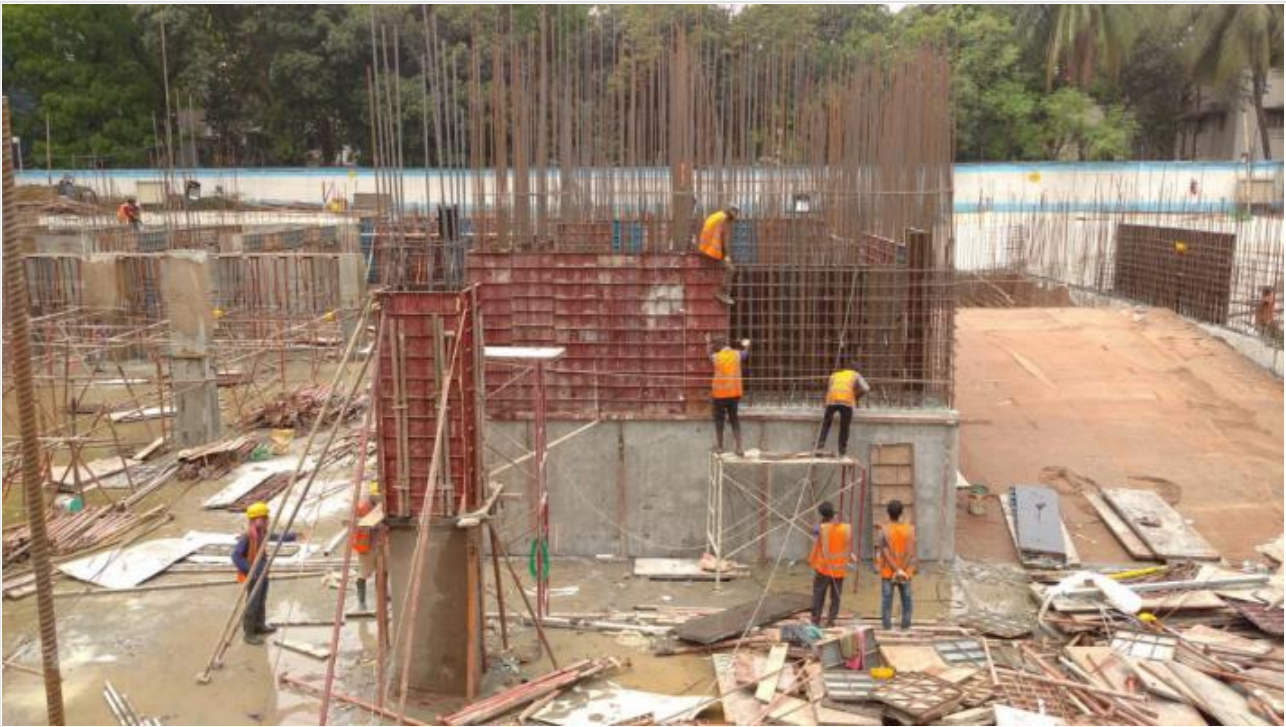
Shear wall shuttering on 23-03-22
