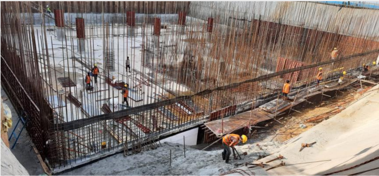
Retaining Wall-North-2nd Lift-Form Work on 10-11-21
