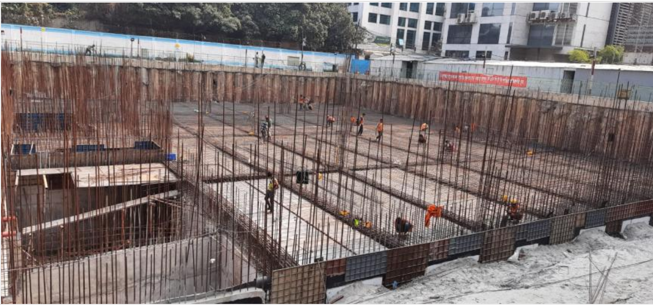
Shuttering and rod binding on 09-01-22
