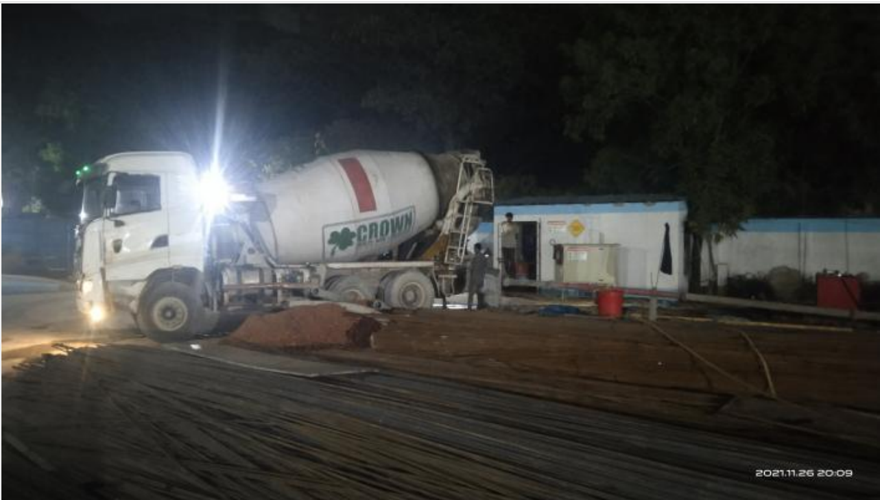
Ready mix concreting on 26-11-21
