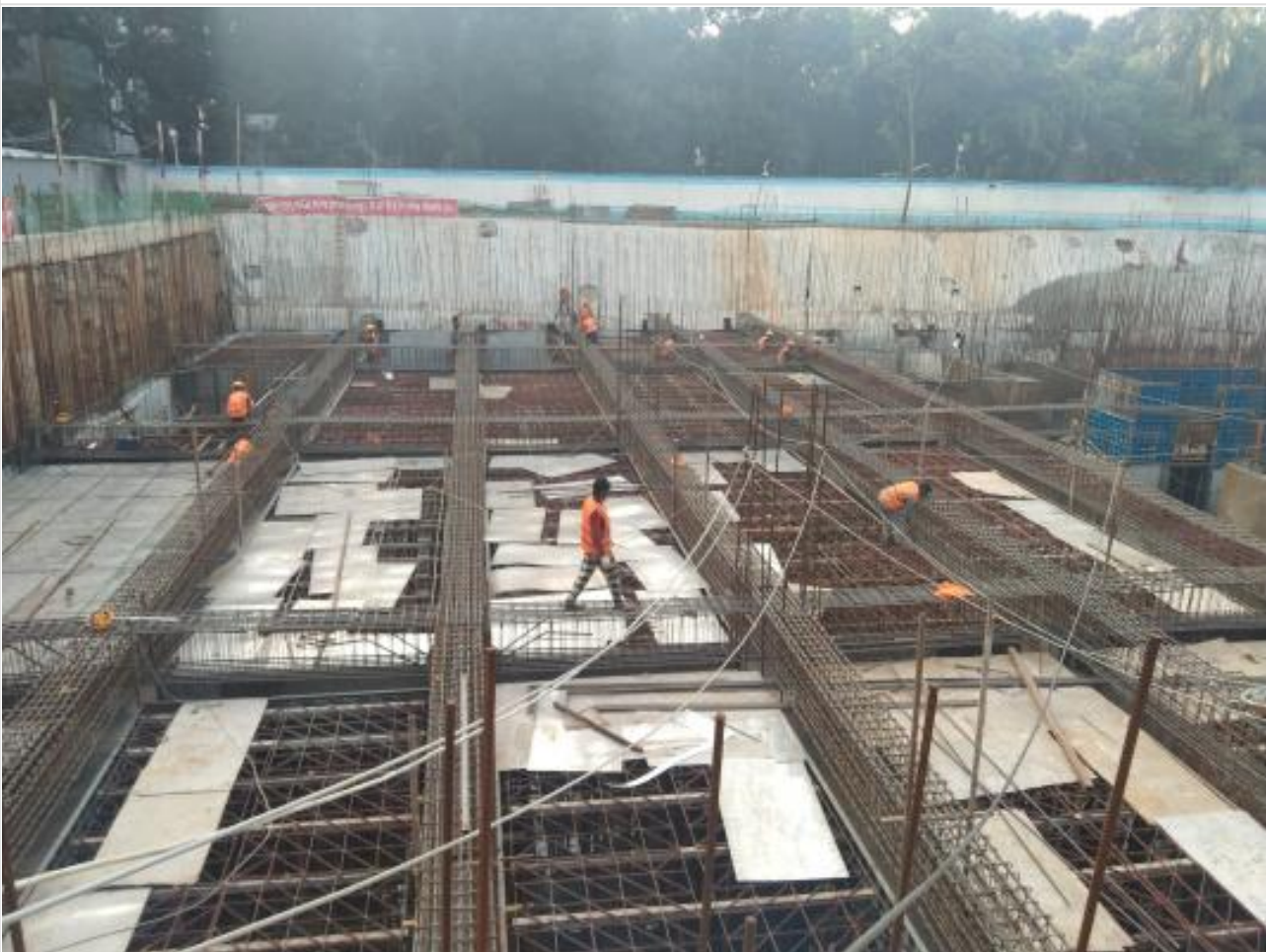
South slab form work and shuttering on 19-12-21
