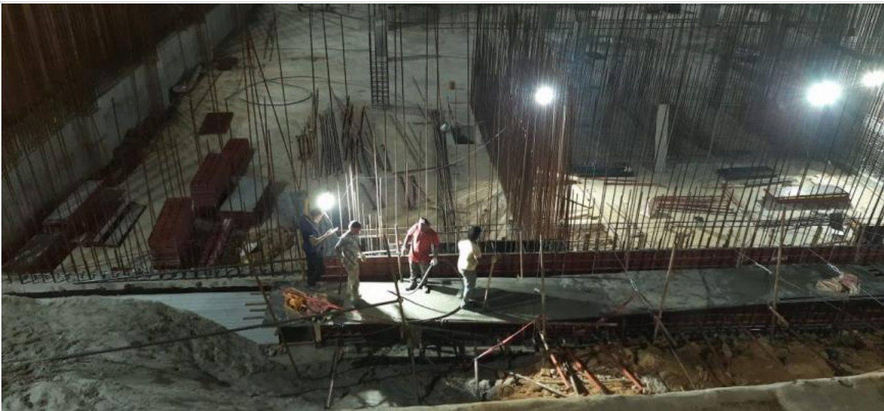
Casting Finish on 05-11-21
