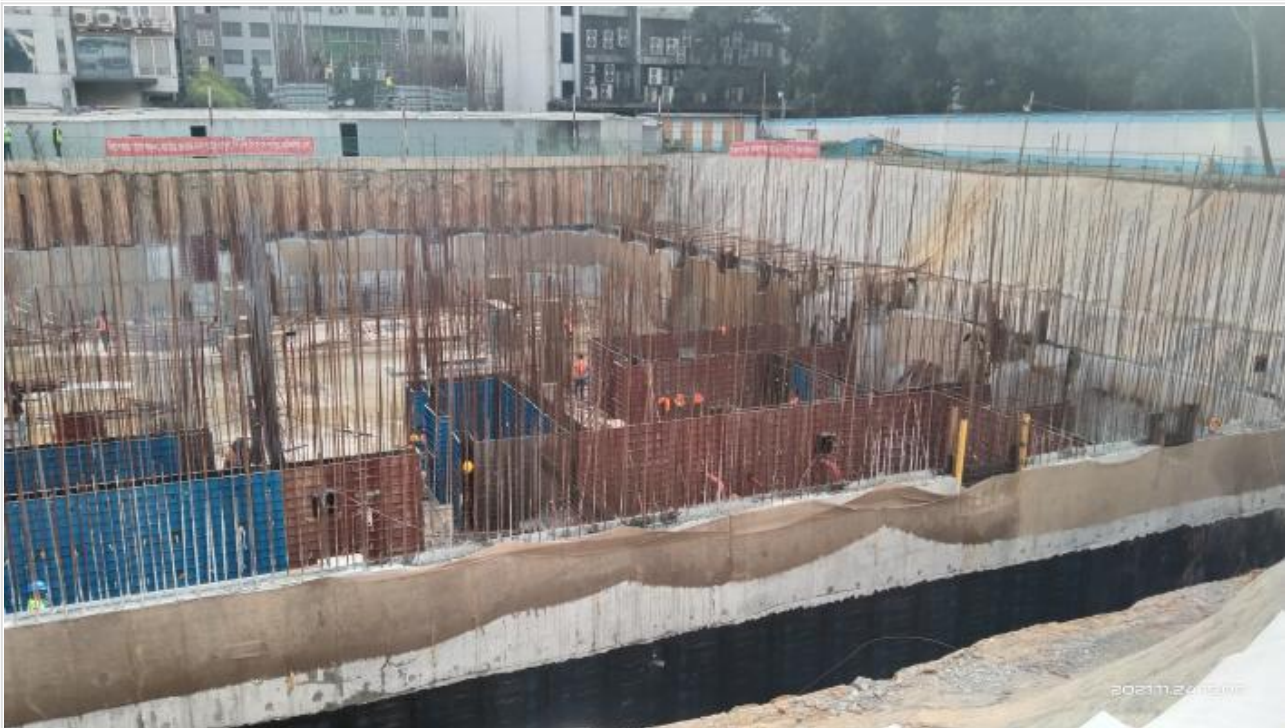
Shear wall and water reserivior shutterin on 24-11-21
