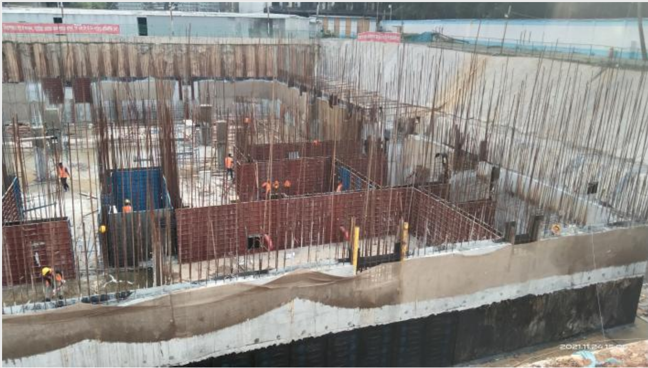
Shuttering work on 24-11-21
