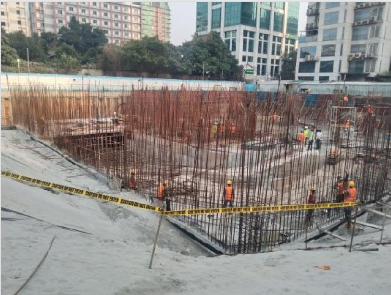
B-1-North retaining wall rebar work on 28-02-22
