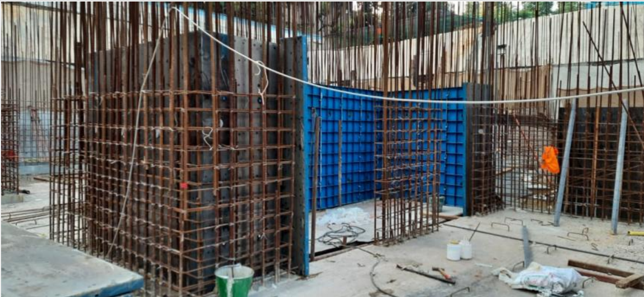
Shear wall shuttering on 21-11-21
