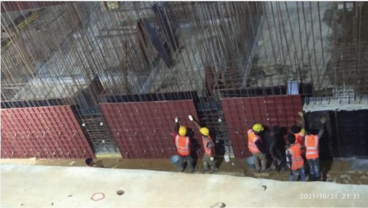
Shuttering work on 31-10-21
