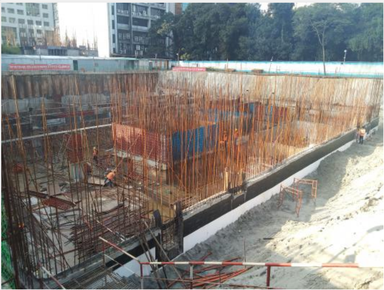
Site picture on 08-12-21
