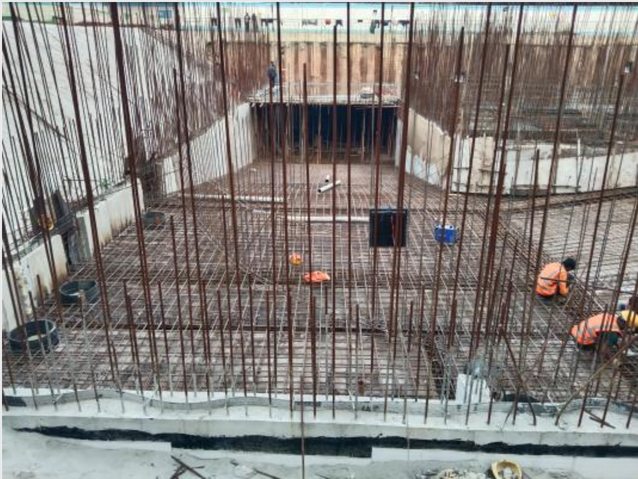
Ramp work on 30-01-22
