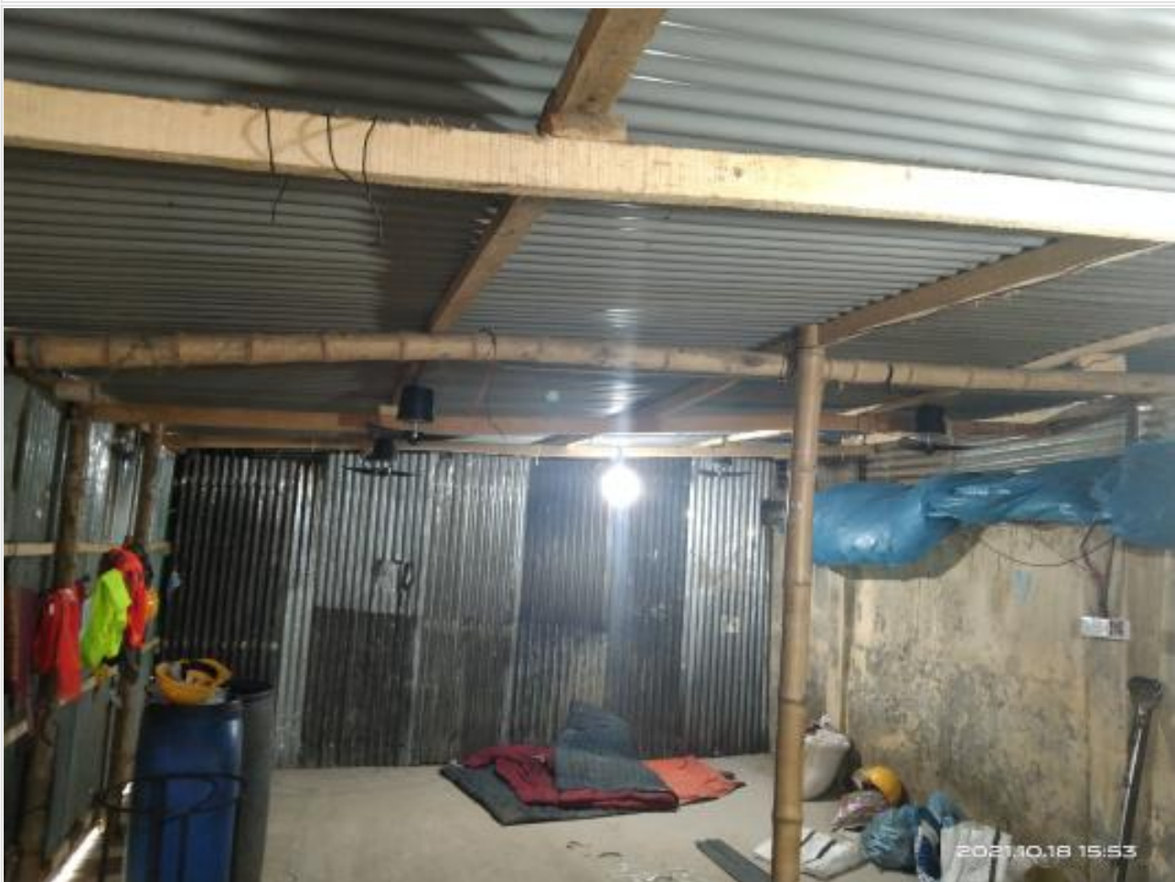
Mobilization work labour shed wiring on 18-10-21
