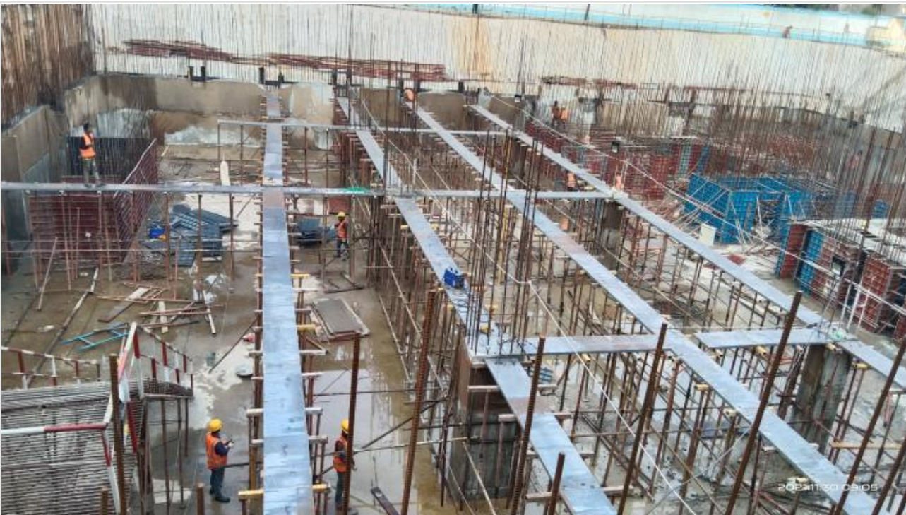
South B1 Slab shuttering on 30-11-21
