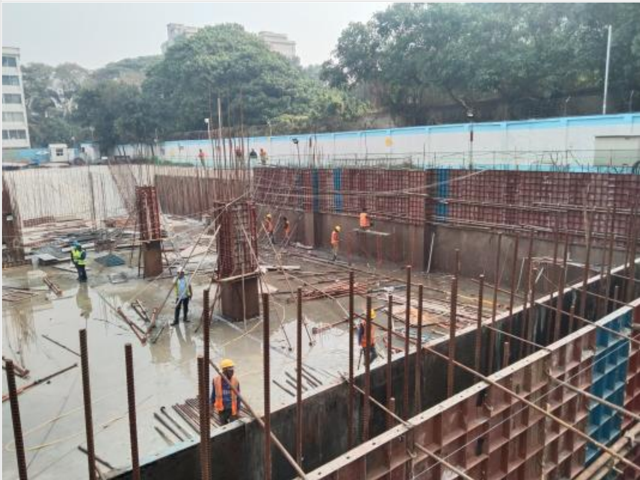
Basement-1-South Column shuttering on 23-02-22
