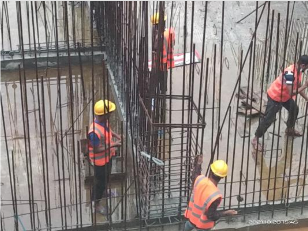
Column ring rod binding on 20-10-21
