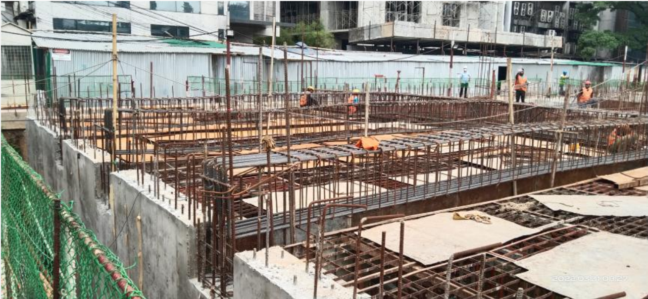
Gr.Floor Slab shuttering and rod binding on 31-03-22
