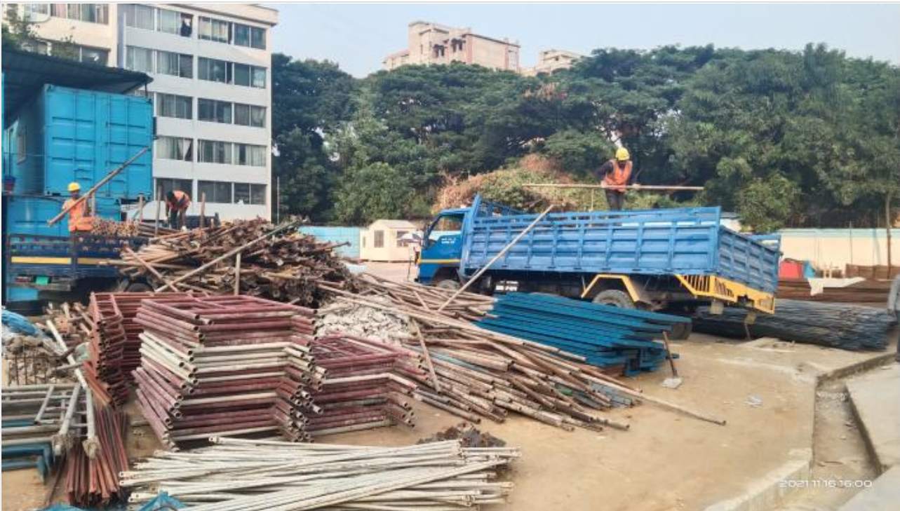
Mobilization slab materials on 16-11-21
