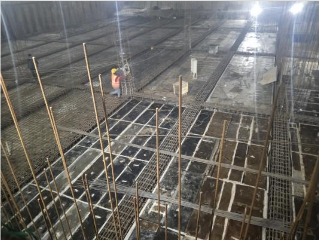
Basement-1-North slab work on 05-01-22
