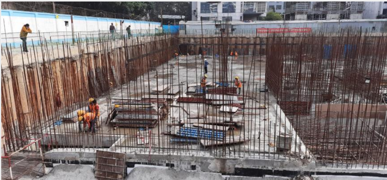
South Retaining wall on 09-02-22
