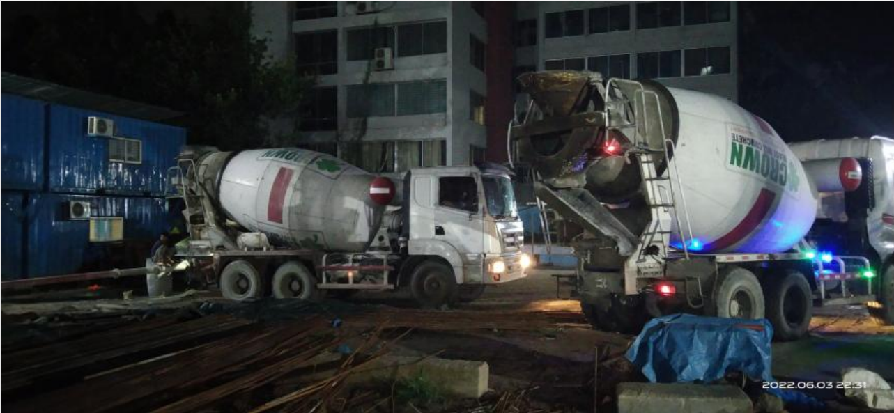
Ready mix car on 03-06-22
