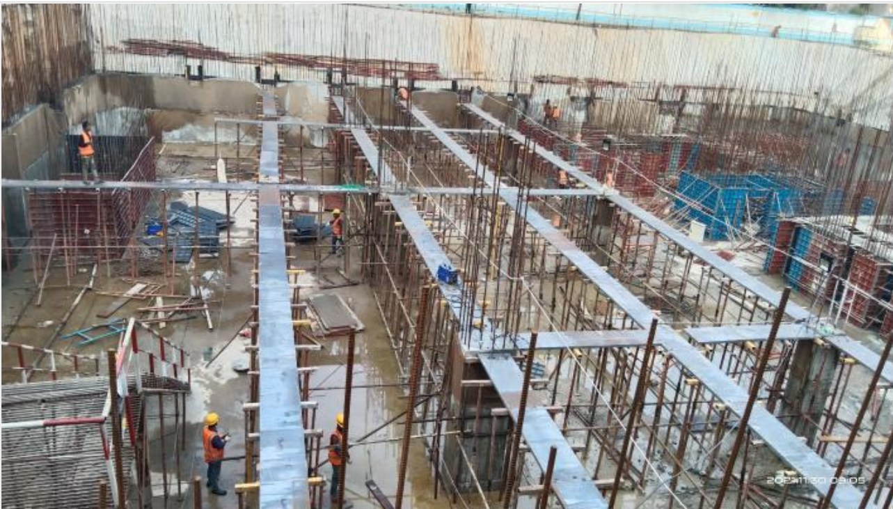
South B1 Slab shuttering on 30-11-21
