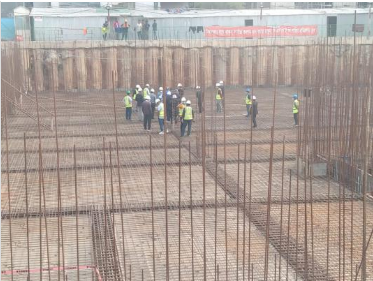
Inspection by American & Local Consultan on 17-01-22
