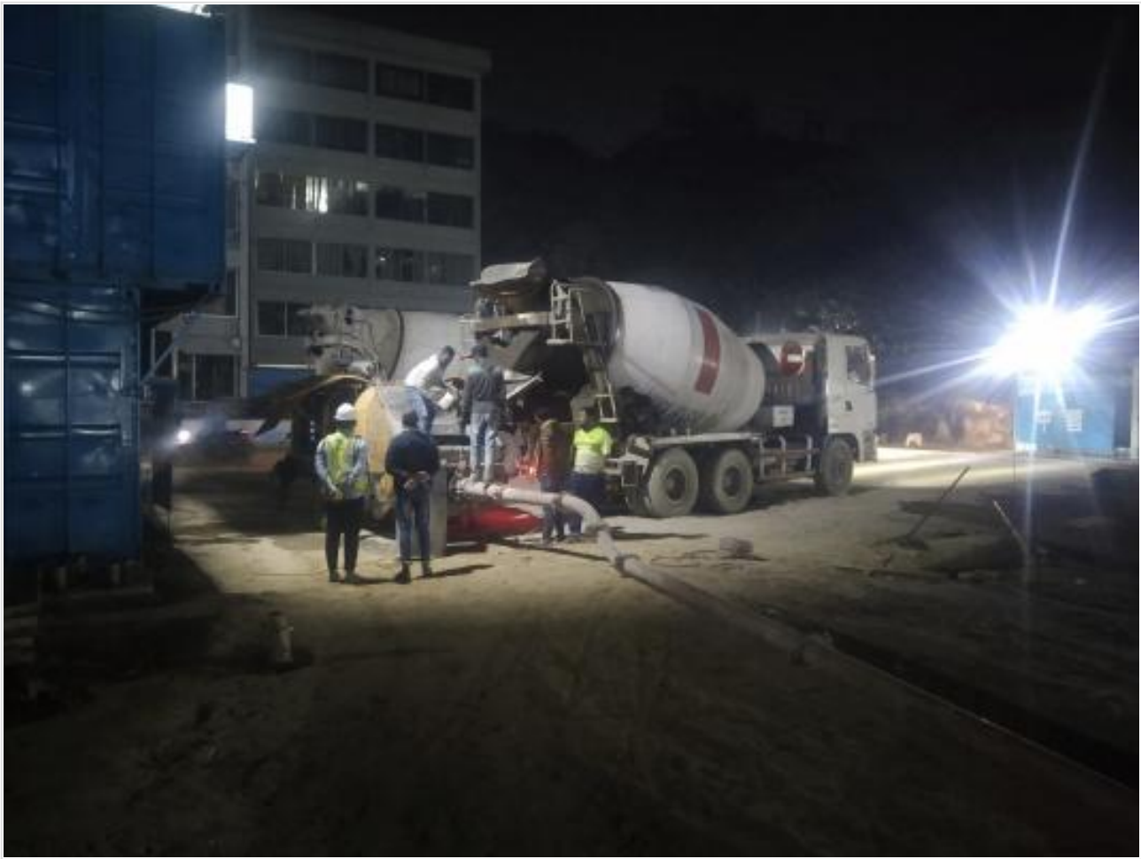
Ready mix on 14-02-22
