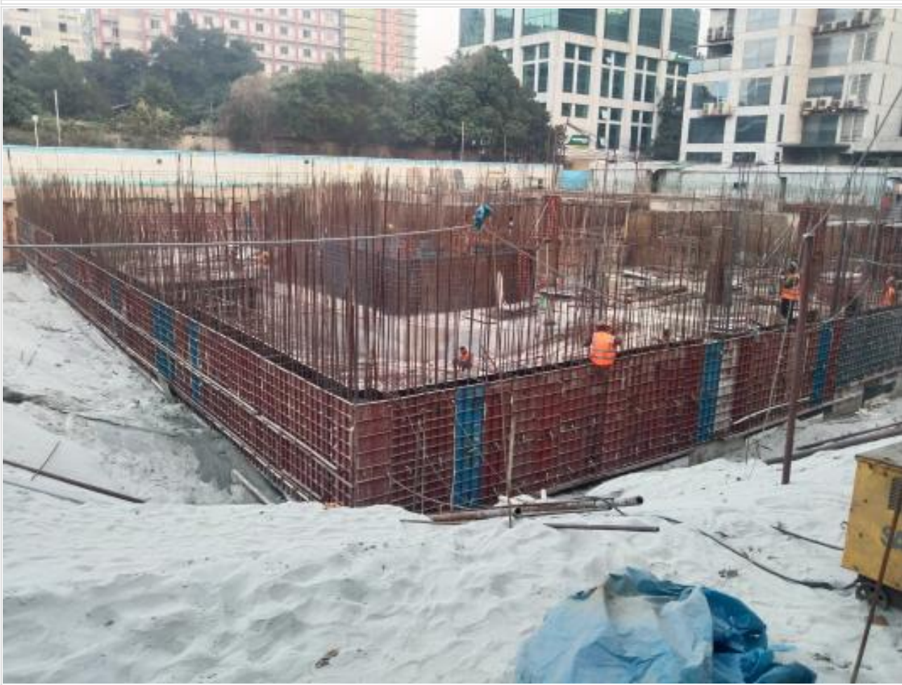
North retaining wall on 07-03-22
