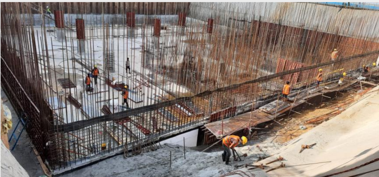
Retaining Wall-North-2nd Lift-Re-bar Wor on 10-11-21
