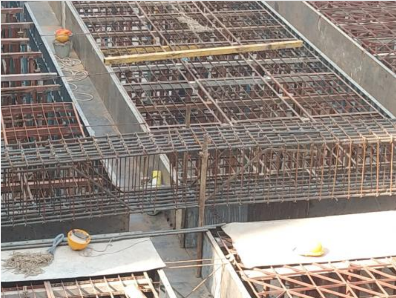
South slab shuttering and rod binding on 15-12-21
