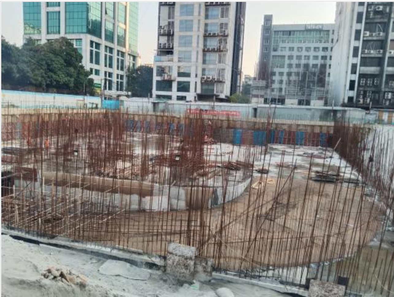
Basement-1-South Retaining wall on 12-02-22
