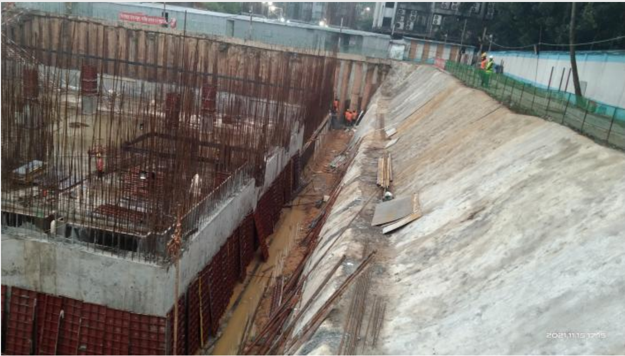
Shuttering work on 15-11-21
