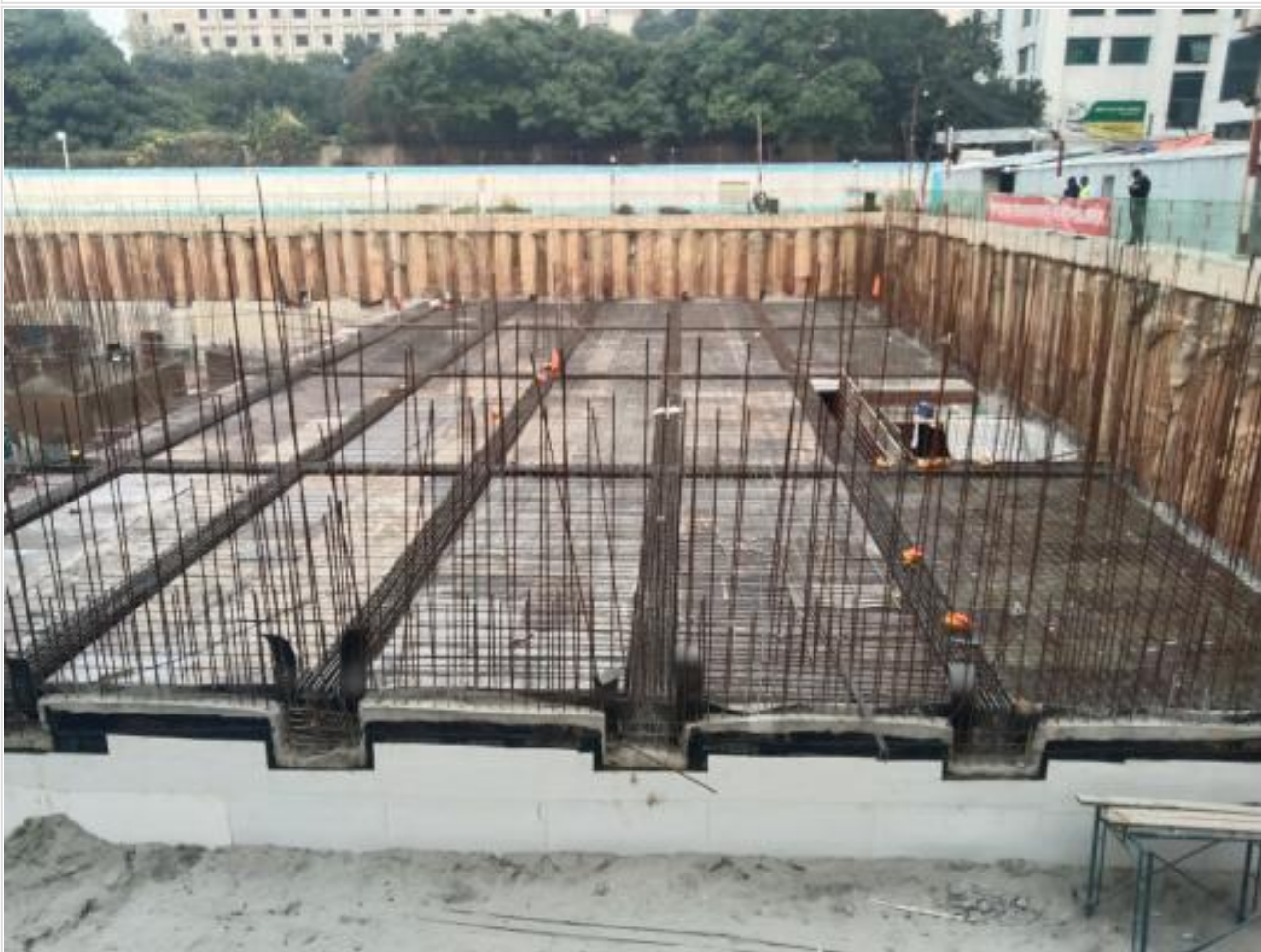
South slab work on 21-12-21
