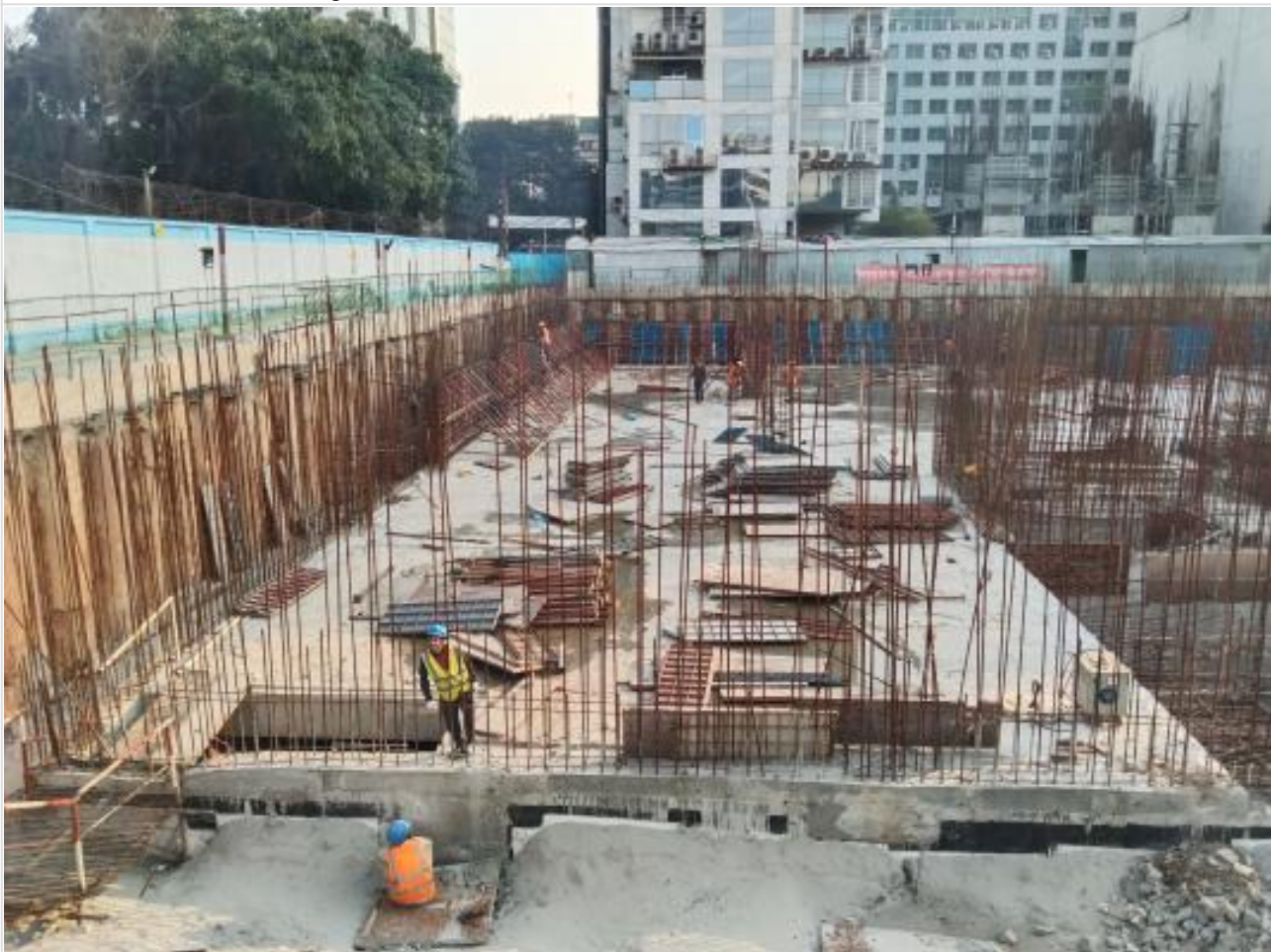
Basement-1-South Retaining Wall-Shutteri on 12-02-22
