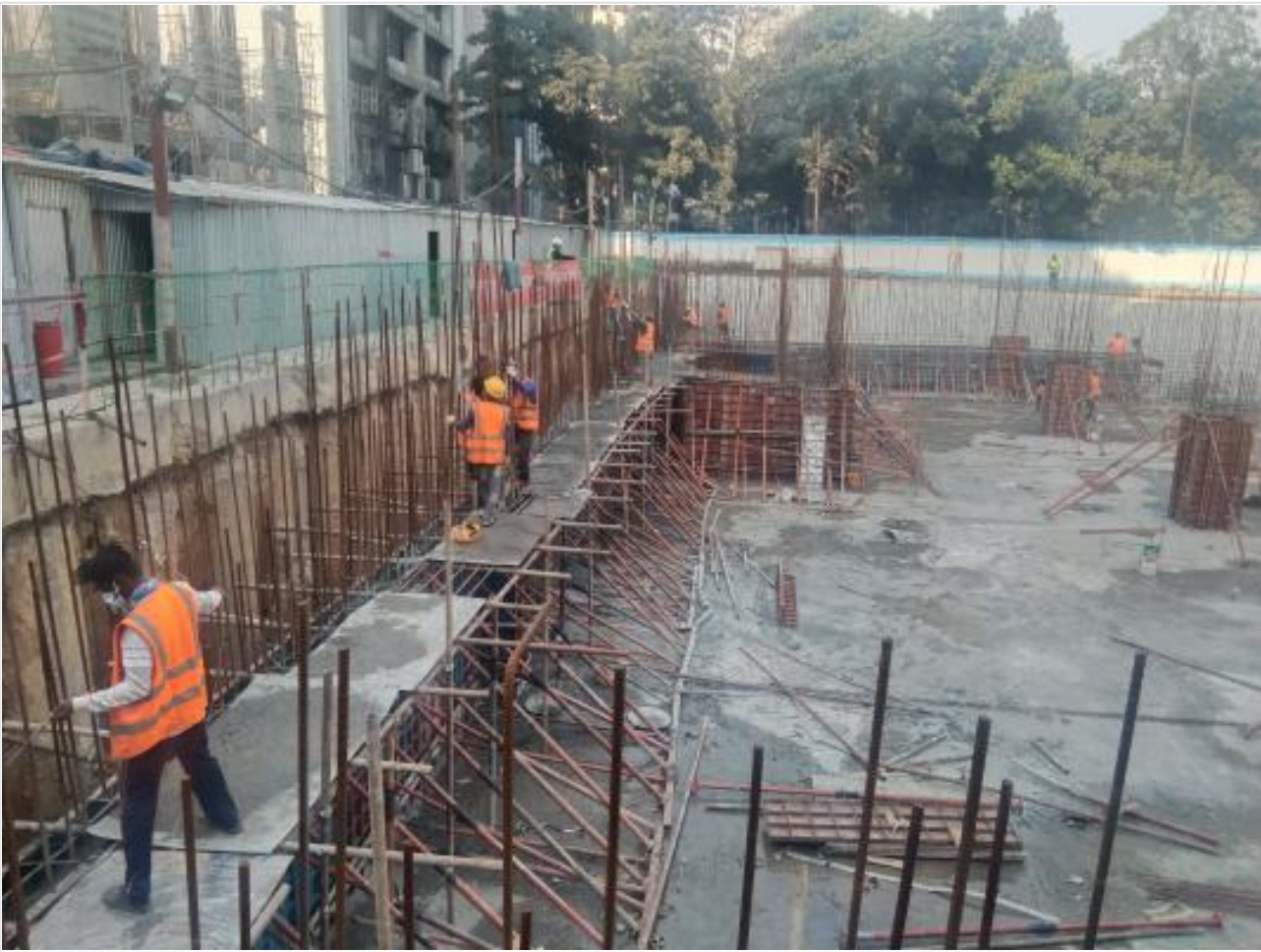
Basement-1-South retaining wall 2nd lift on 16-02-22
