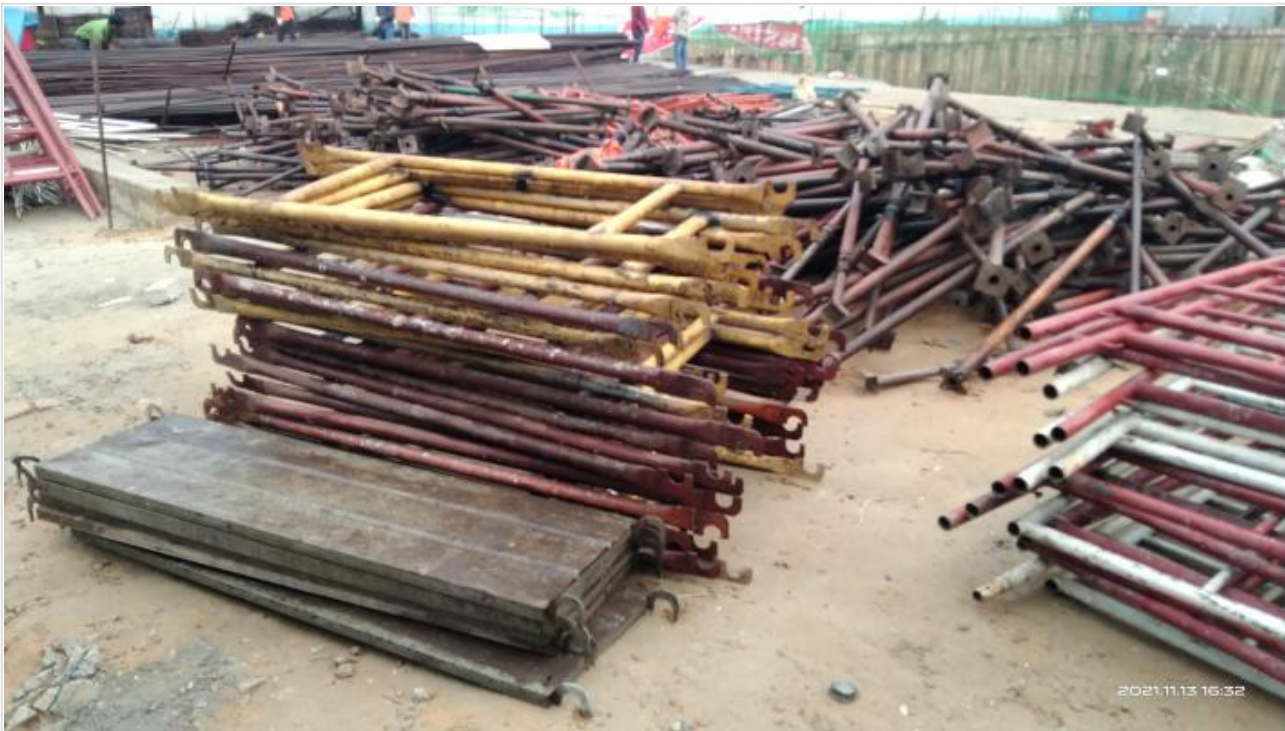
Scaffolding Bumper on 13-11-21
