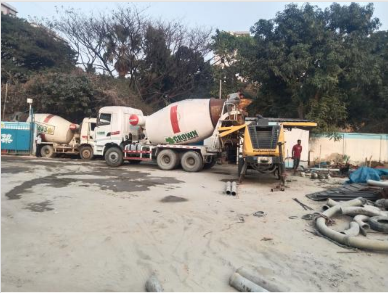
Ready-mix Concrete Truck and Pump on 26-02-22
