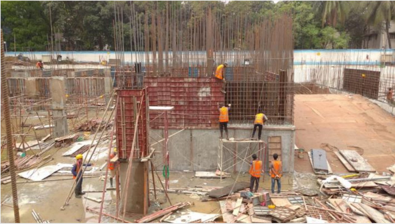
Shear wall shuttering on 23-03-22
