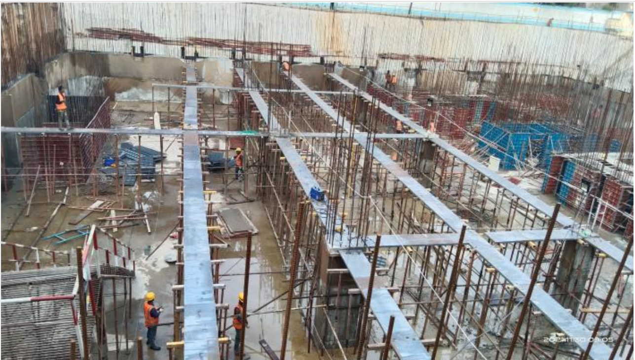
South B1 Slab shuttering on 30-11-21
