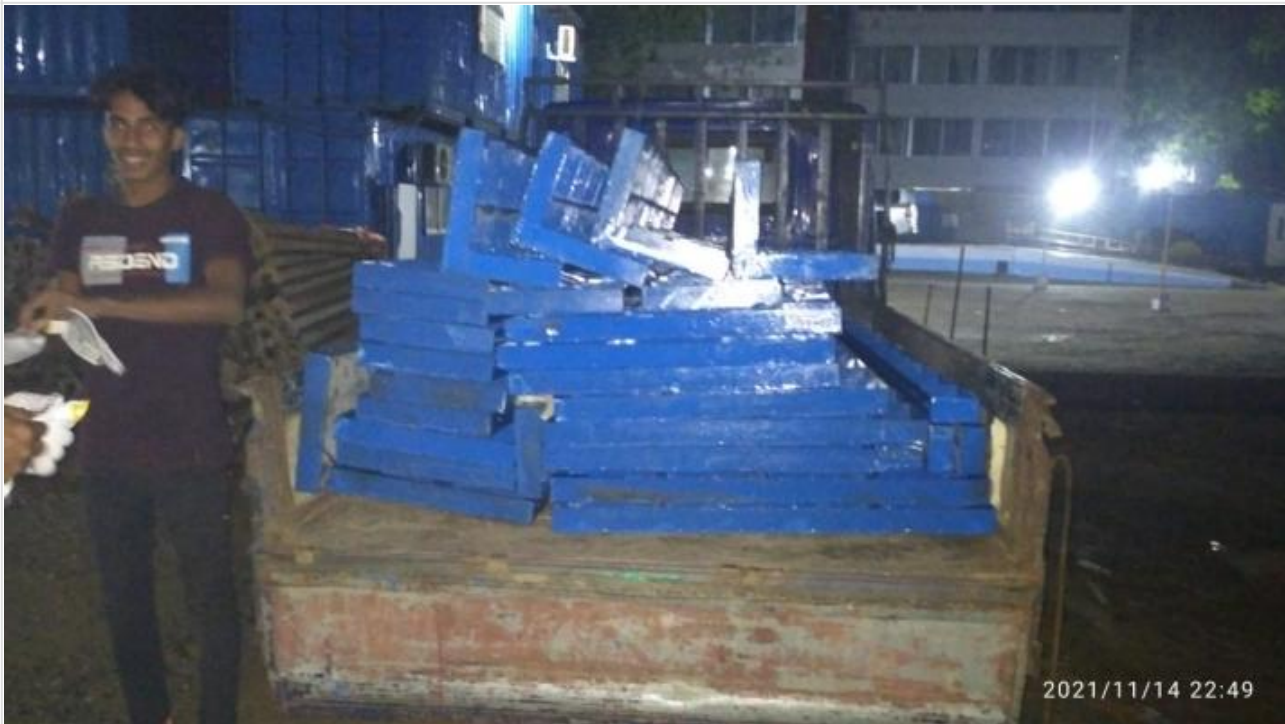
Shear wall shutter on 14-11-21
