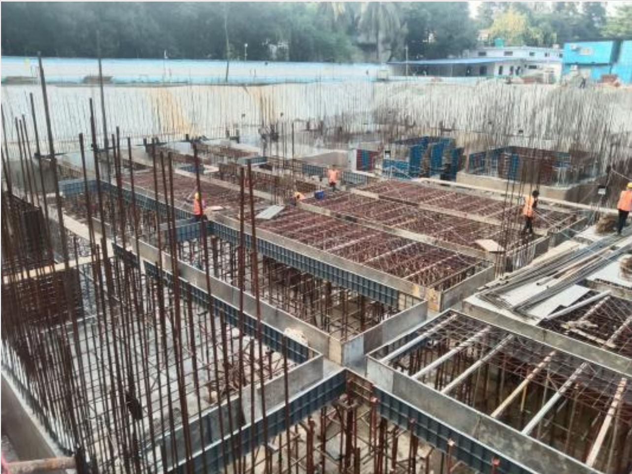
B1 south slab shuttering on 13-12-21
