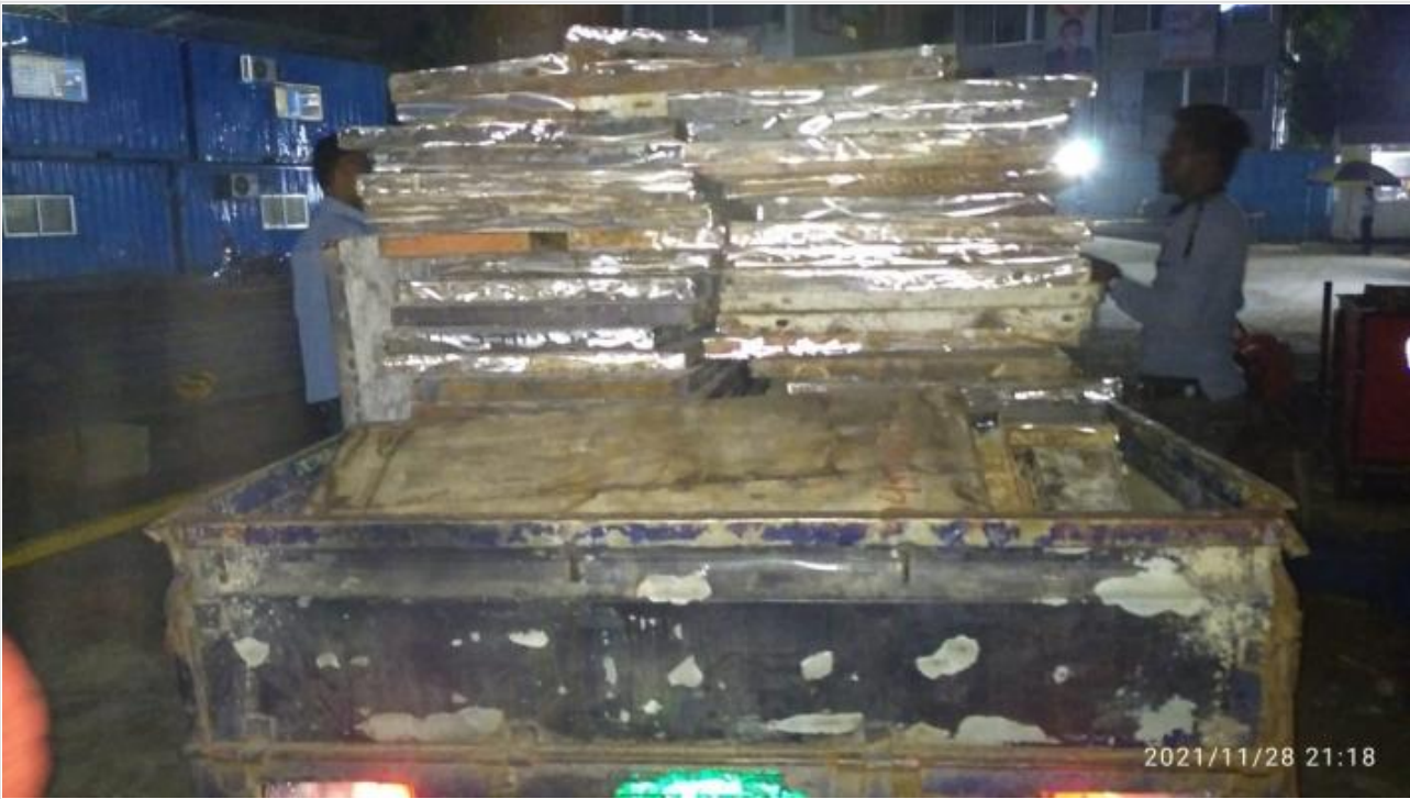
Slab south shutter mobilization on 28-11-21
