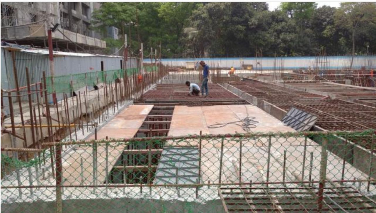
Slab shuttering on 23-03-22
