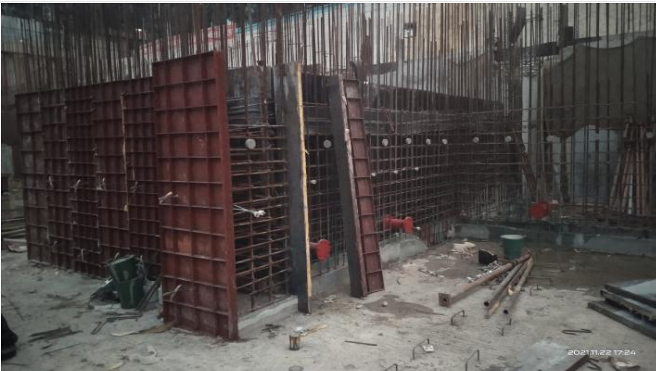
Water tank shuttering on 22-11-21
