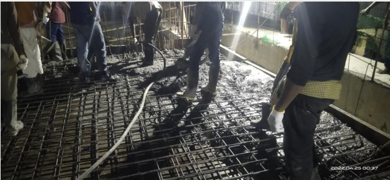
Ground Floor Slab concreting on 24-04-22
