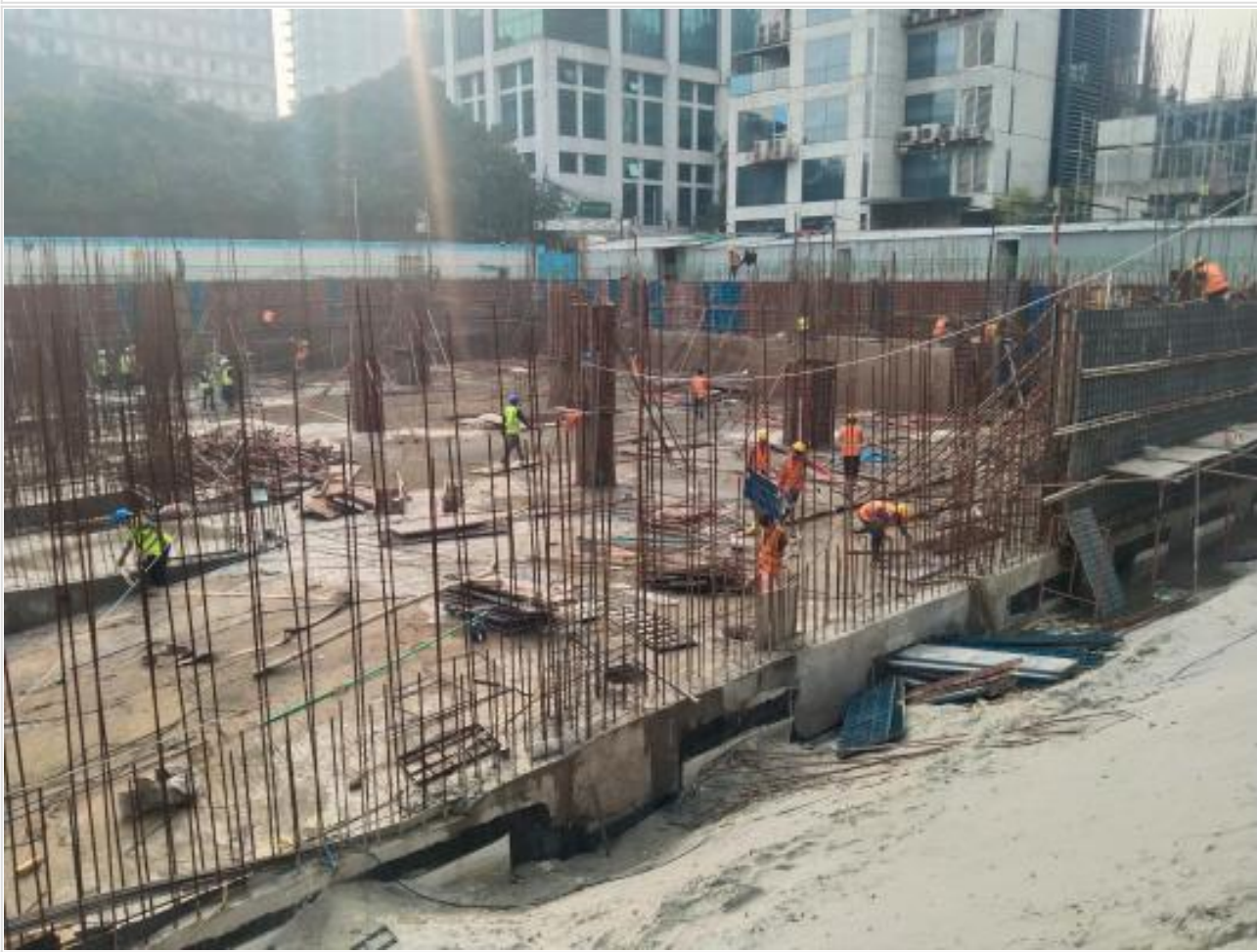
Basement-1-South retaining wall on 23-02-22
