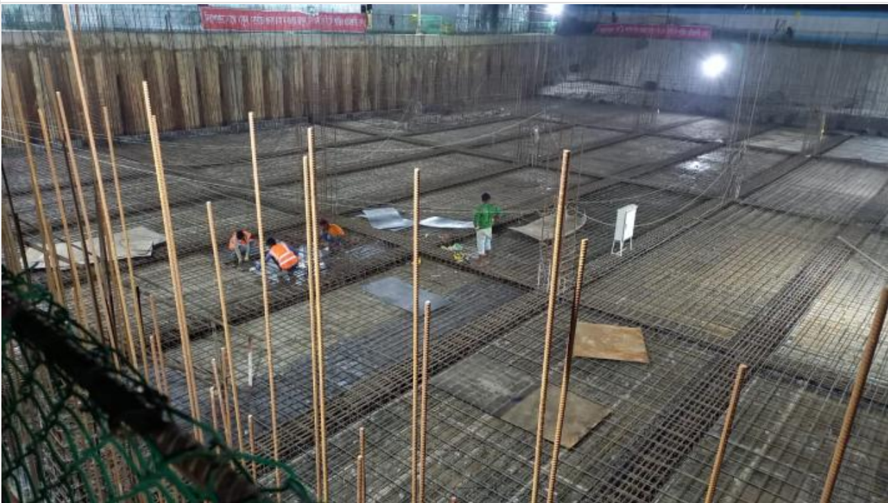
Shuttering work on 09-01-22
