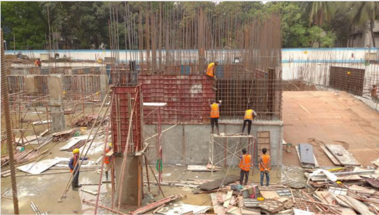
Shear wall shuttering on 23-03-22
