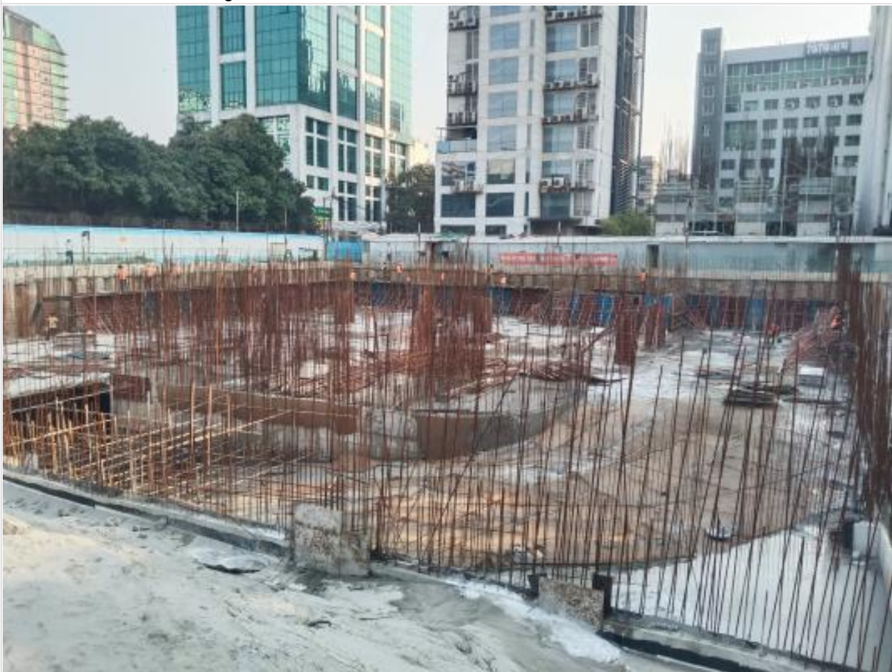
Basement-1-south retaining wall-Re-bar on 16-02-22
