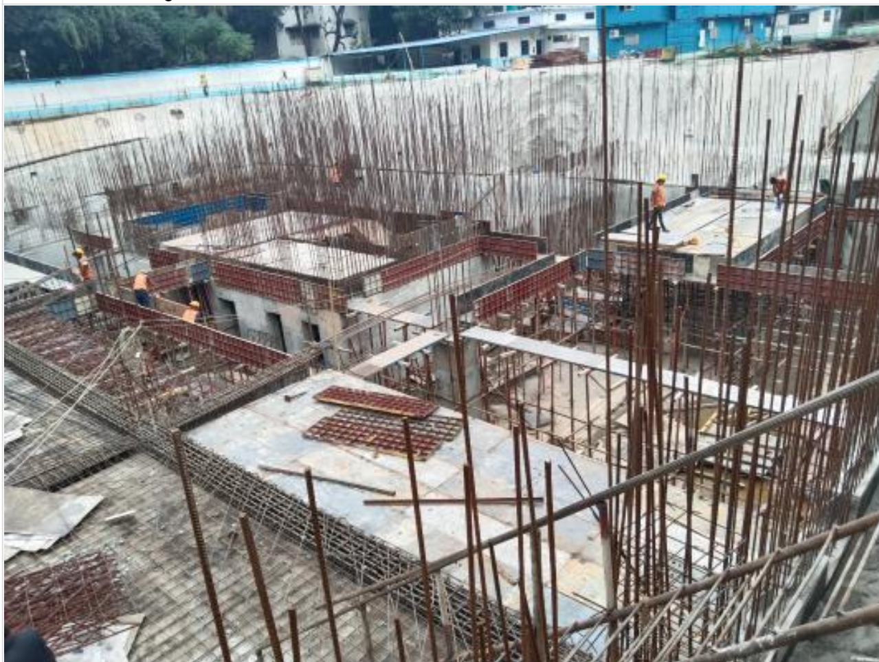
North slab shuttering on 29-12-21
