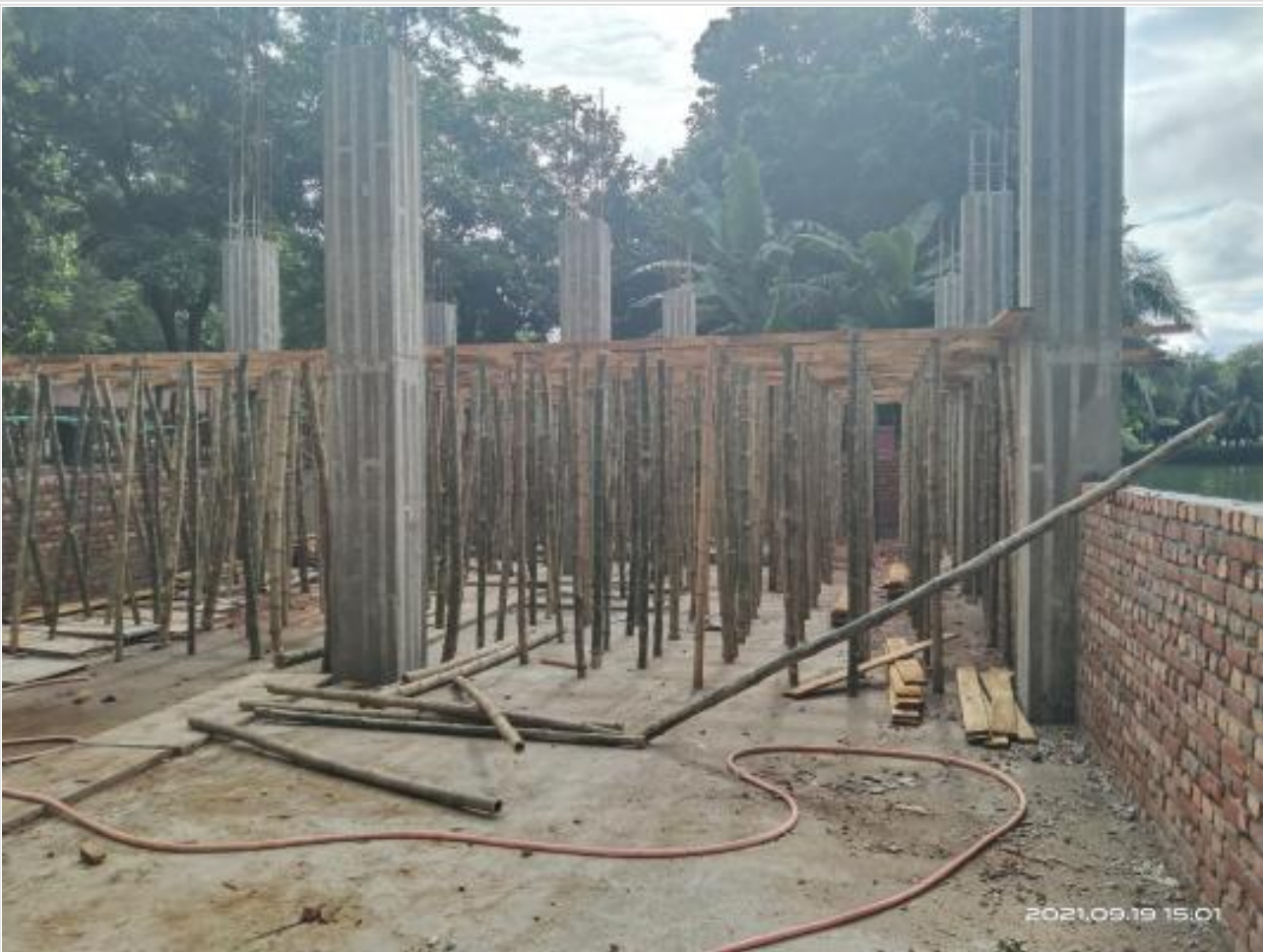
Fire Tank CC work on 19-09-21
