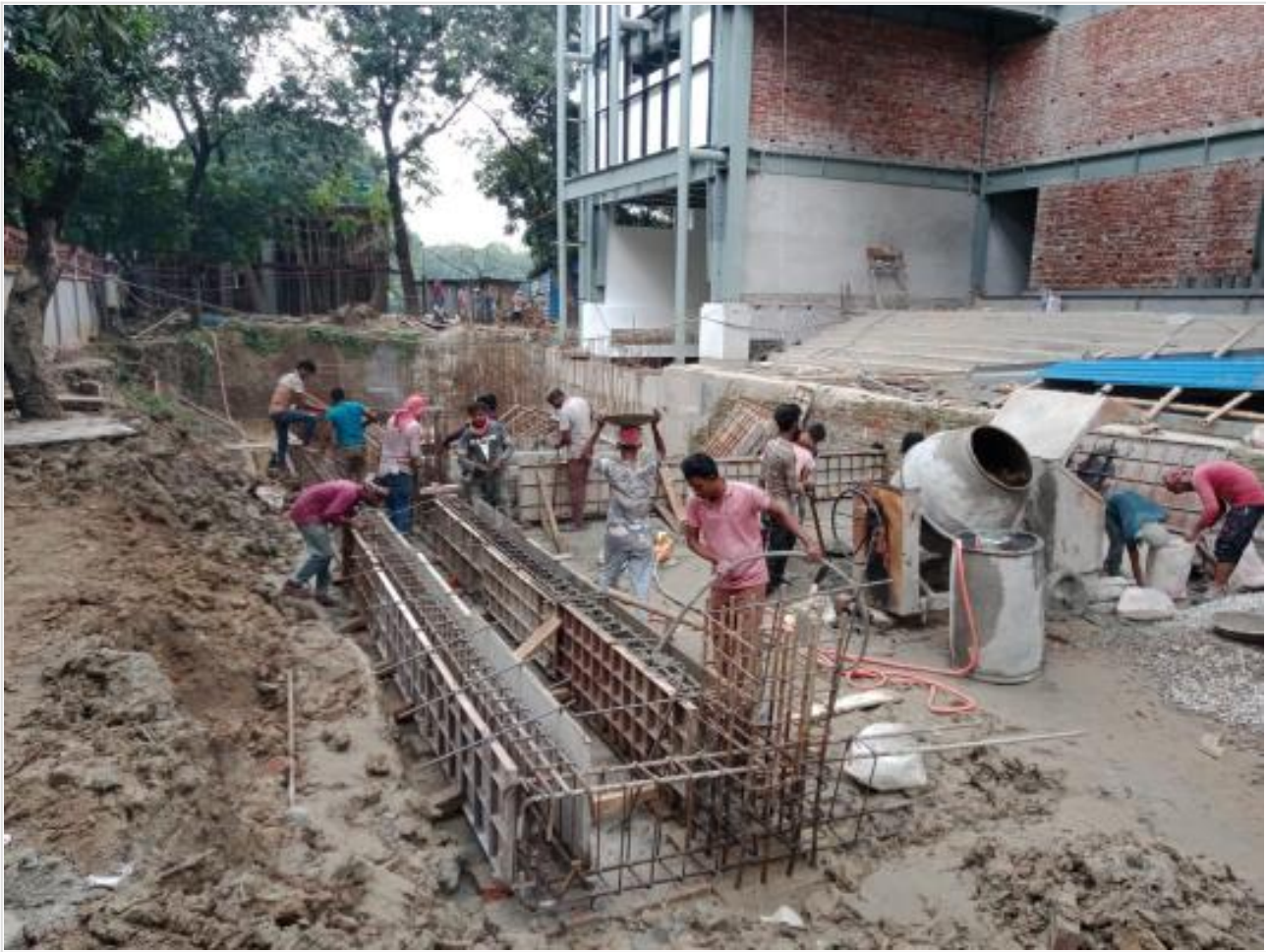
South canopy GB casting on 14-10-21
