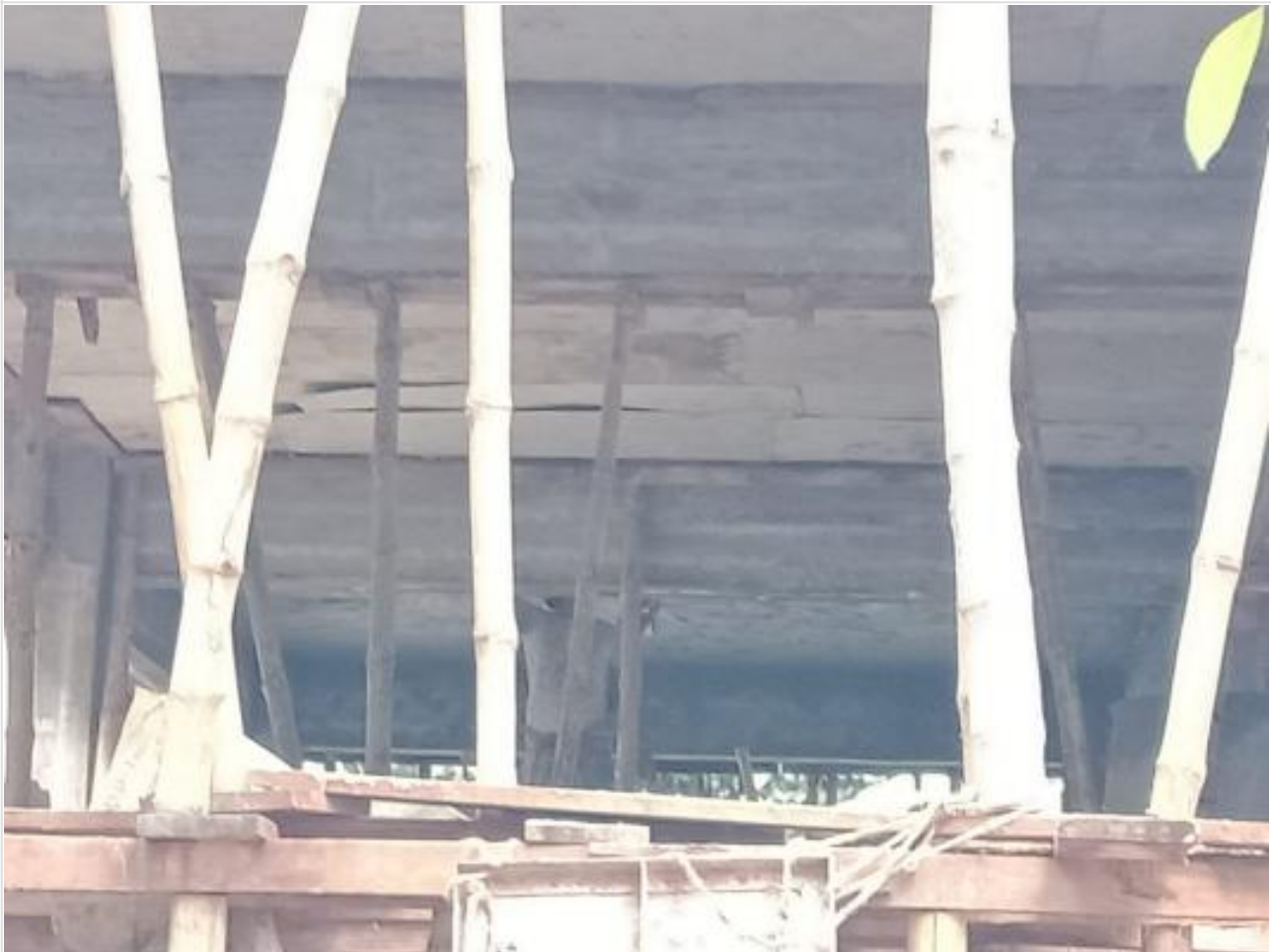
Generator Room shutter remove on 20-10-21
