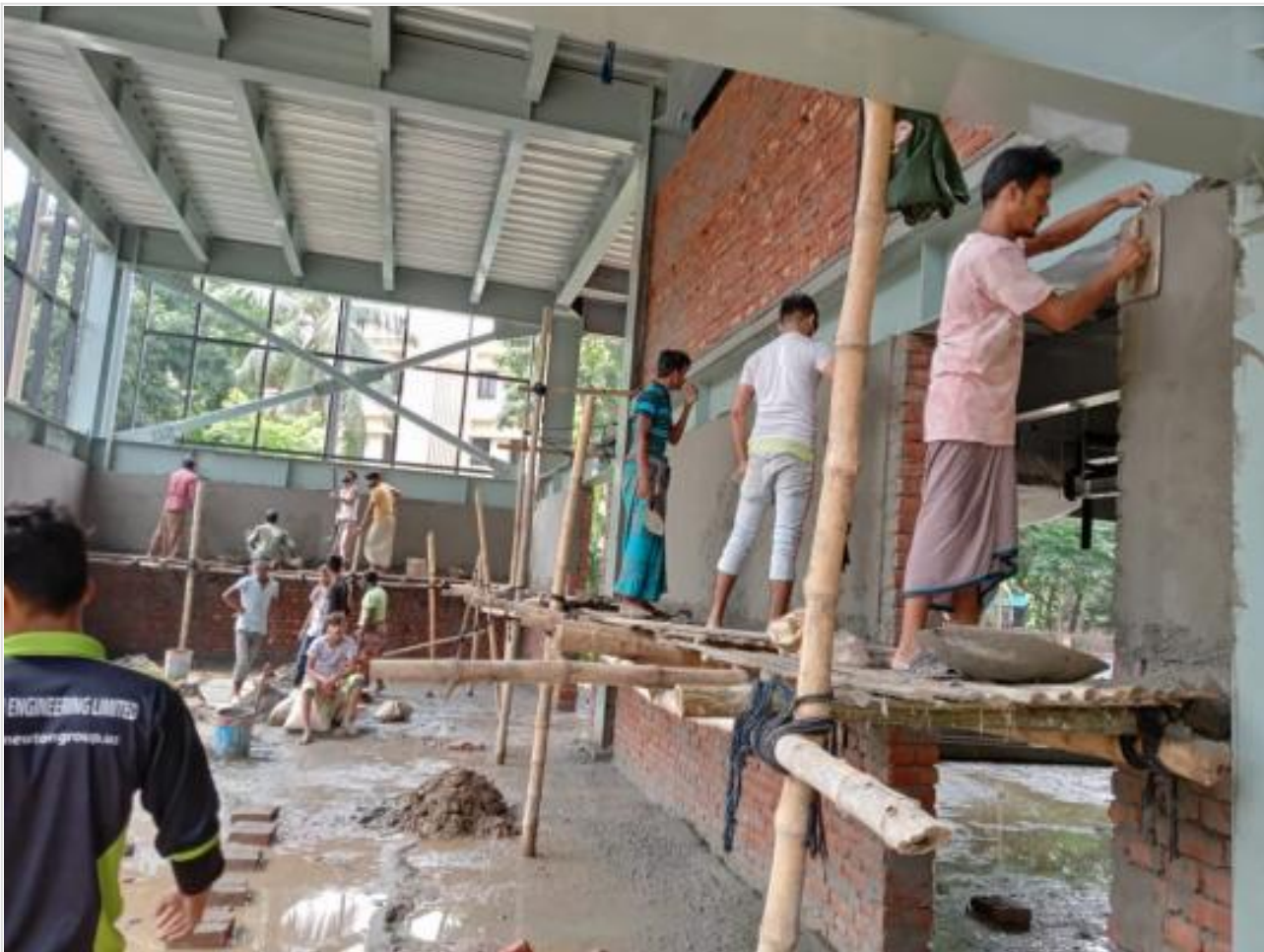
GF Mezzanine Shear Wall Plasteing on 09-08-21
