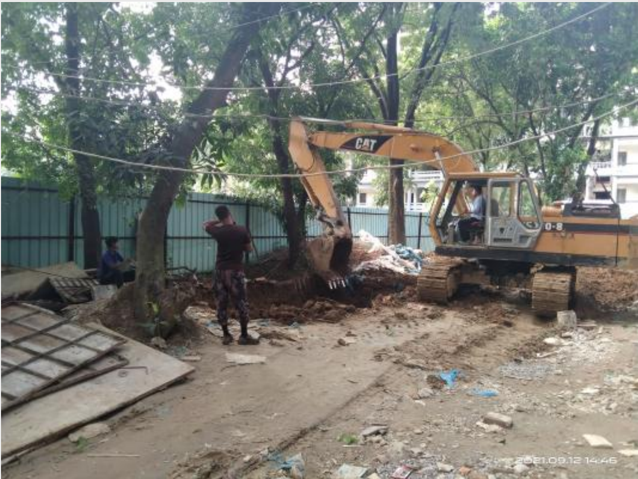
Earth excavation work for septic tank on 12-09-21
