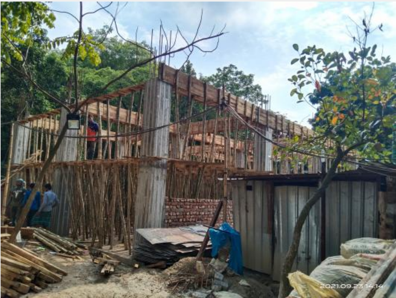
Generator room shuttering work on 23-09-21
