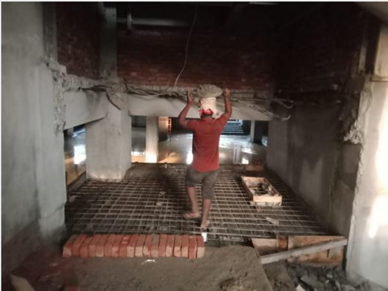
MDB room slab casting on 15-09-21
