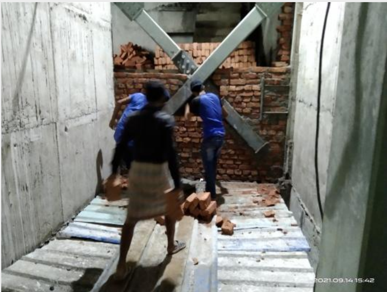
Brick work for lift on 14-09-21
