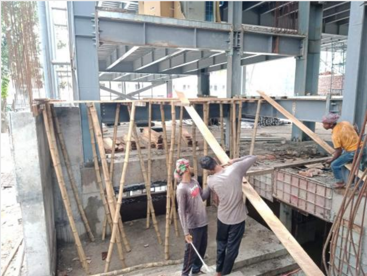
Ground Floor-Stair Shuttering on 04-06-21
