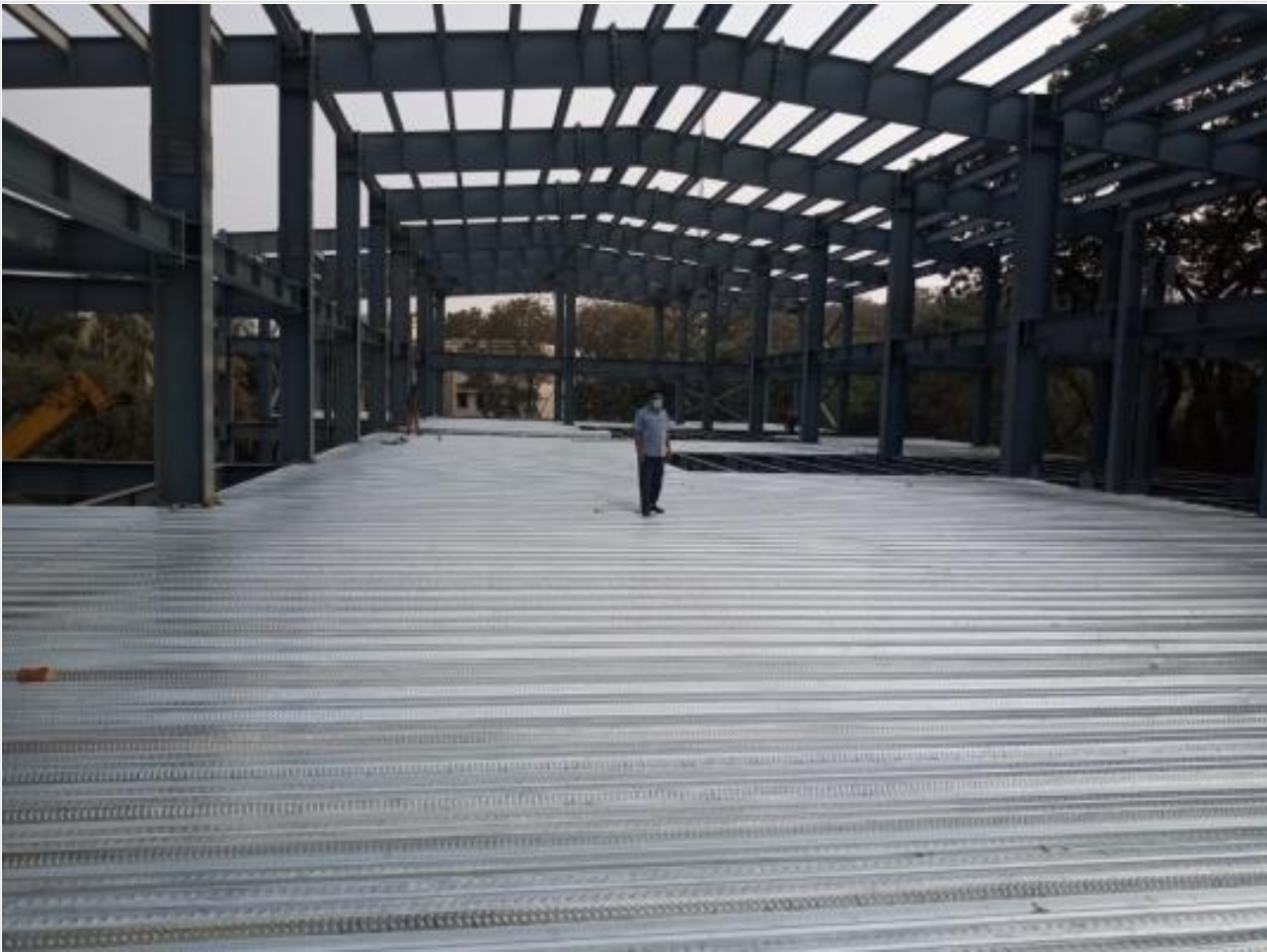
Decking Slab installation on 22-03-21
