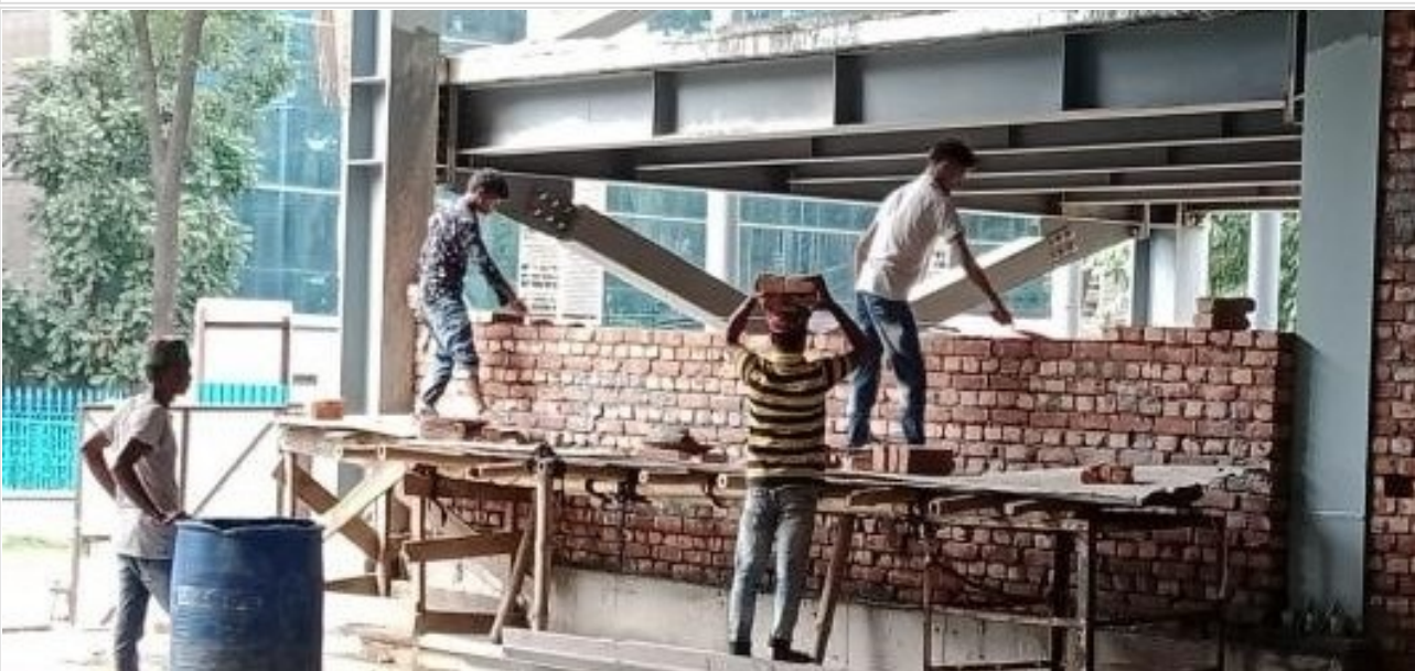
Ground Floor Brick Work on 19-05-21
