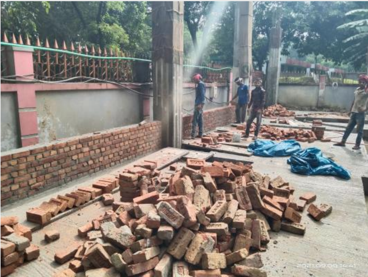
Generator room brick work on 09-09-21
