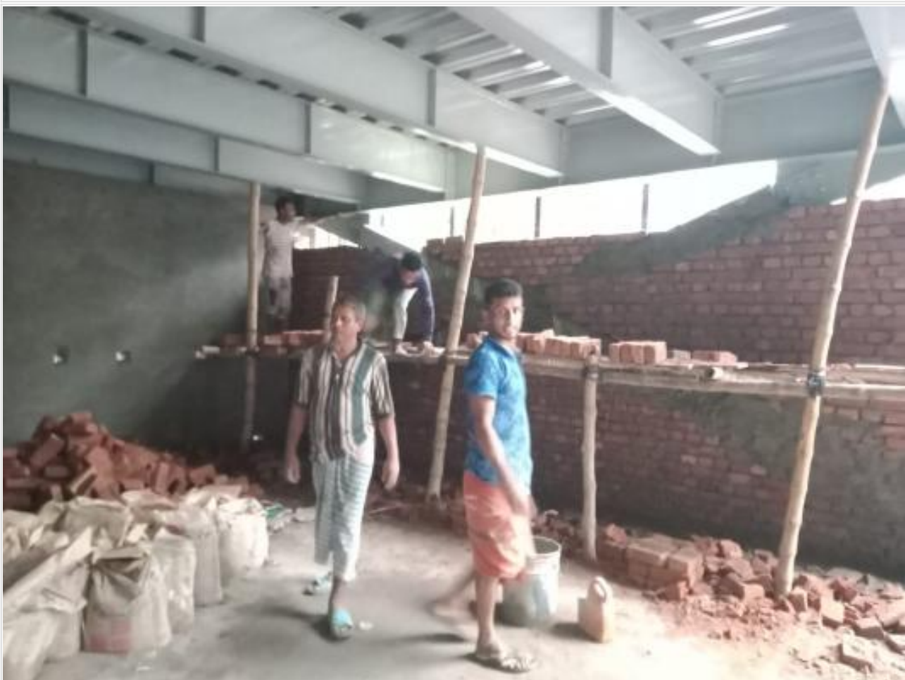
GF brick work on 10-08-21
