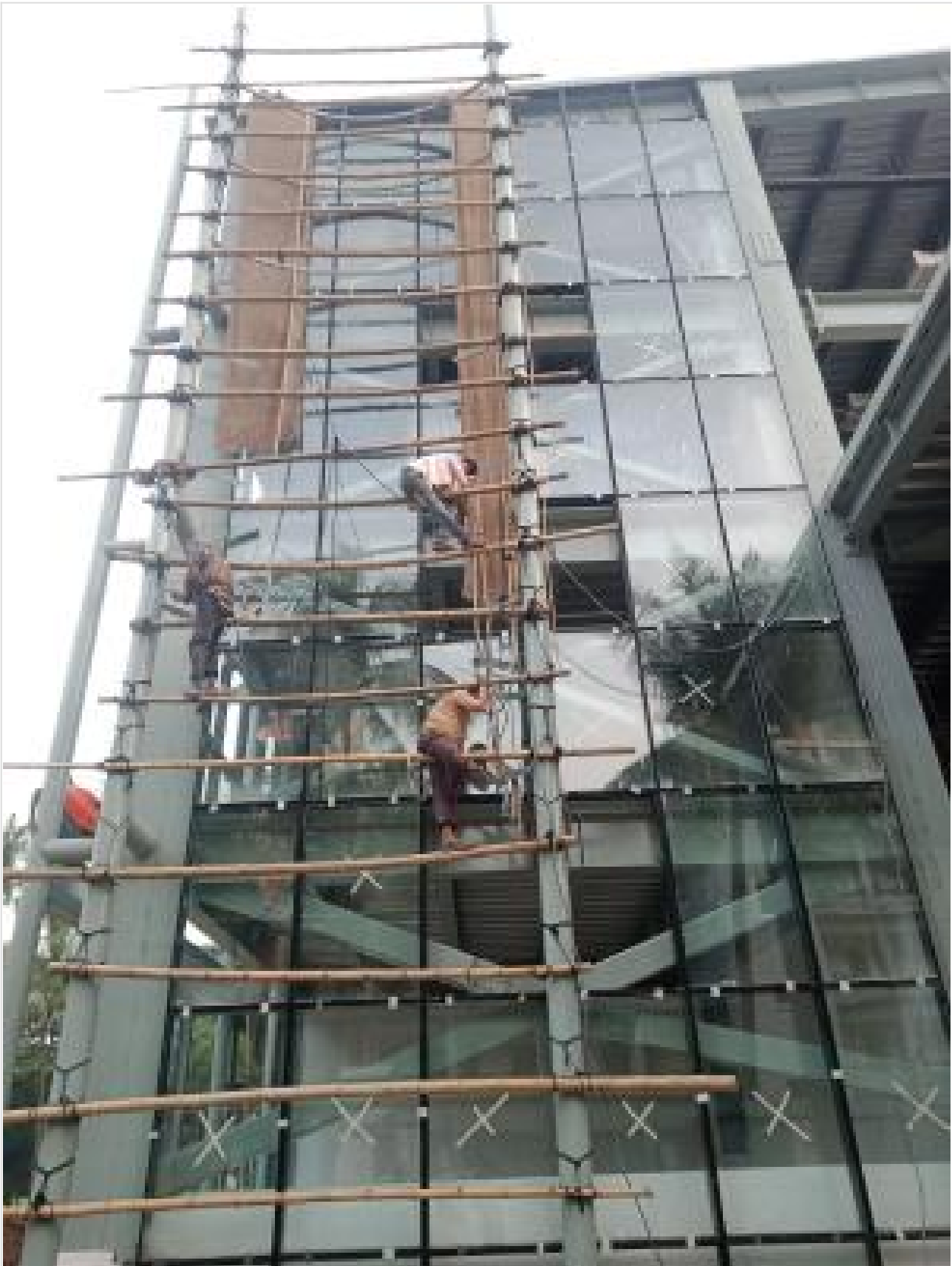
ACP angle frame setting on 11-10-21
