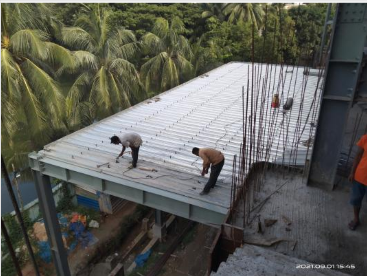
East Canopy Roofing work on 01-09-21
