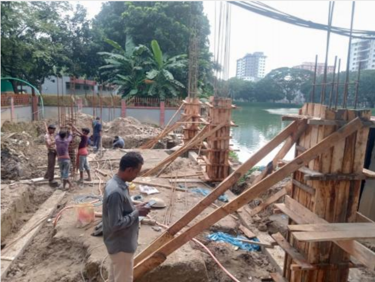
Generator room column casting on 14-08-21
