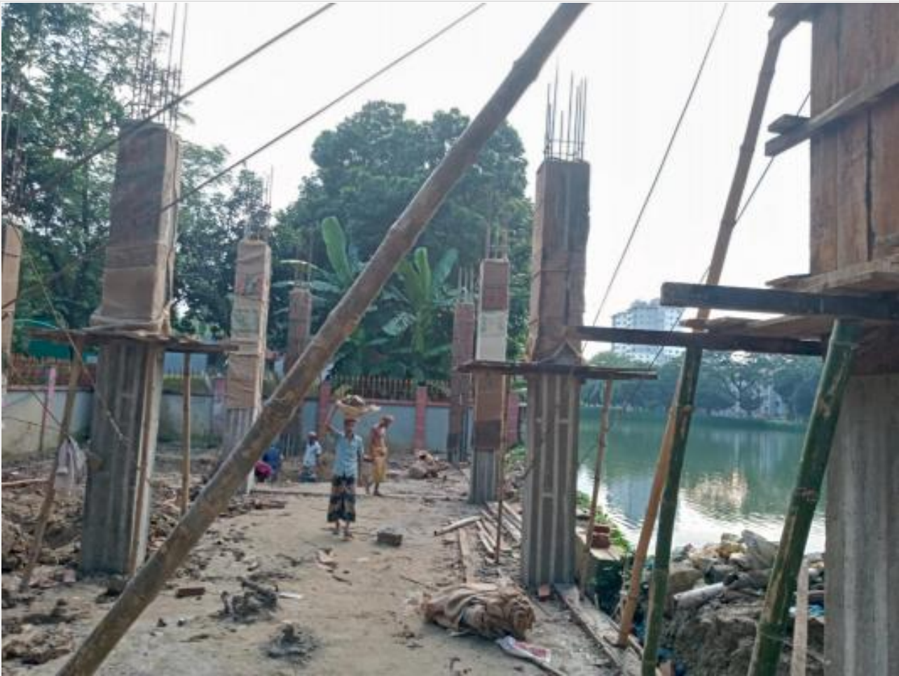
Generator room column shuttering on 27-08-21
