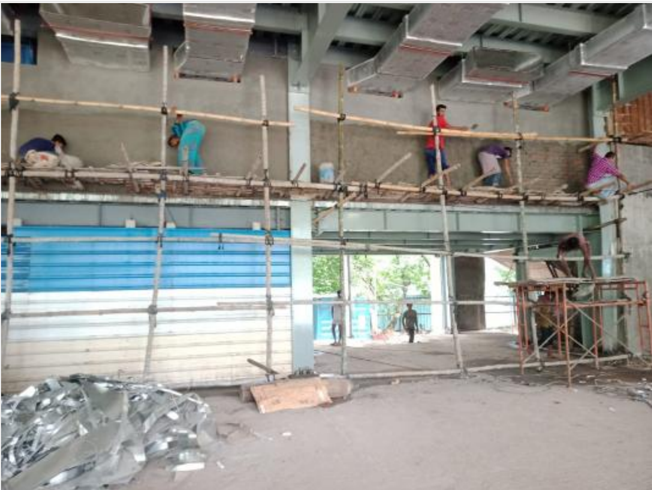
Ground Floor Mezzanine Plastering on 06-08-21
