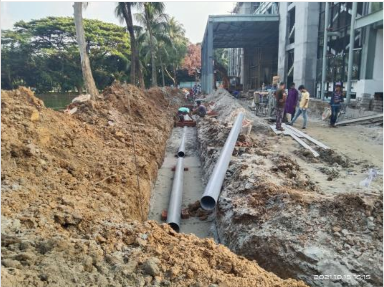
Under ground uPVC pipe line work on 15-10-21
