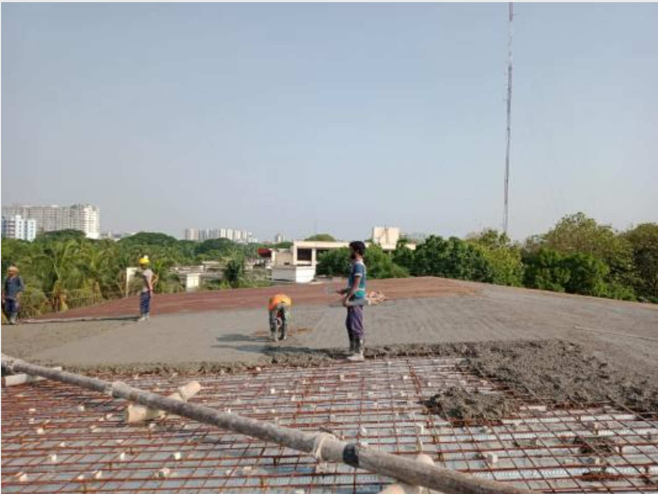
Roof Slab Concreting on 06-05-21
