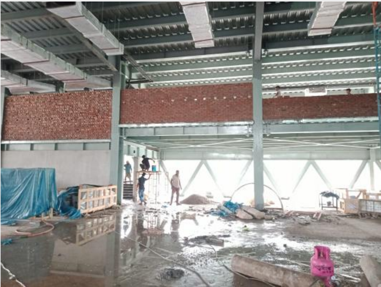
FFM Brick work on 05-10-21
