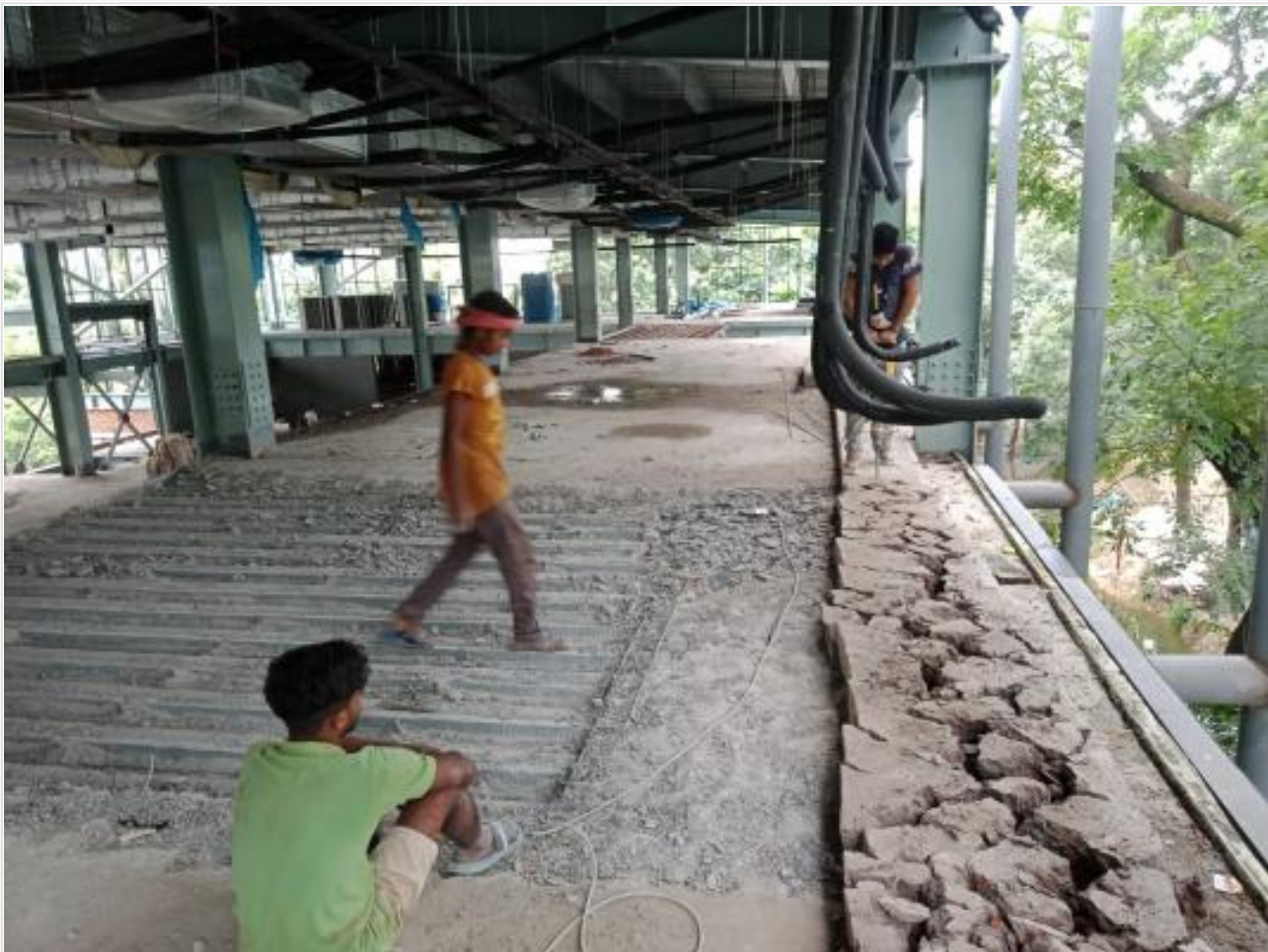
FF Mezzanine dismantling work on 20-08-21
