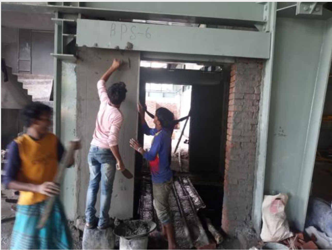
Lift door wall plaster on 22-09-21
