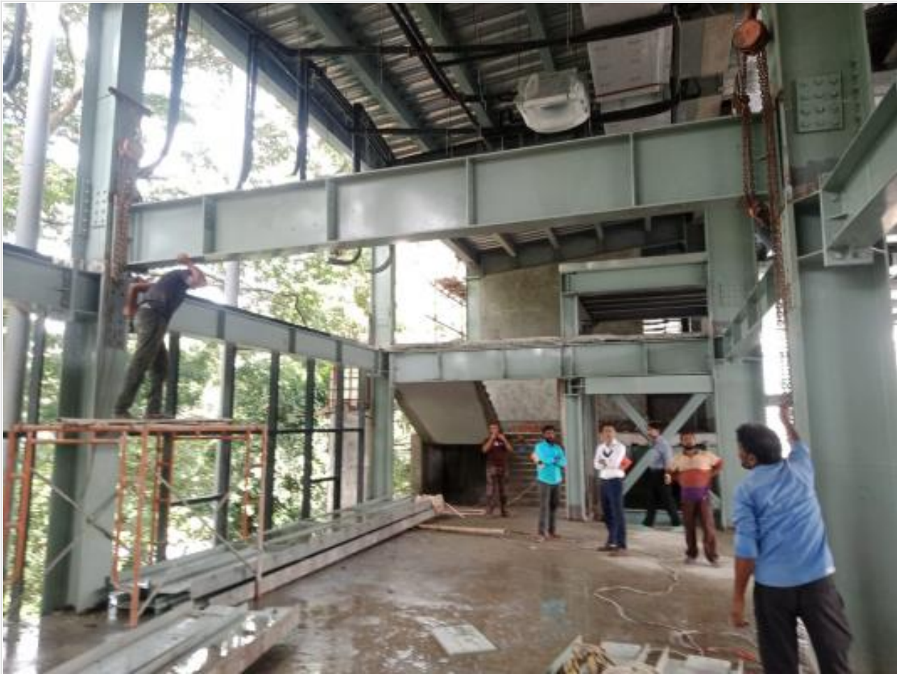
FF Mezzanine floor re-construction on 06-09-21
