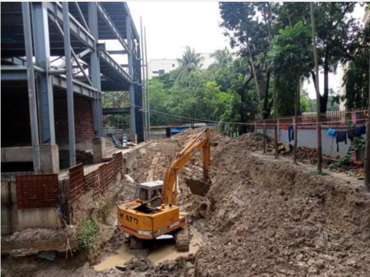
Fire water reservoir excavation on 07-06-21
