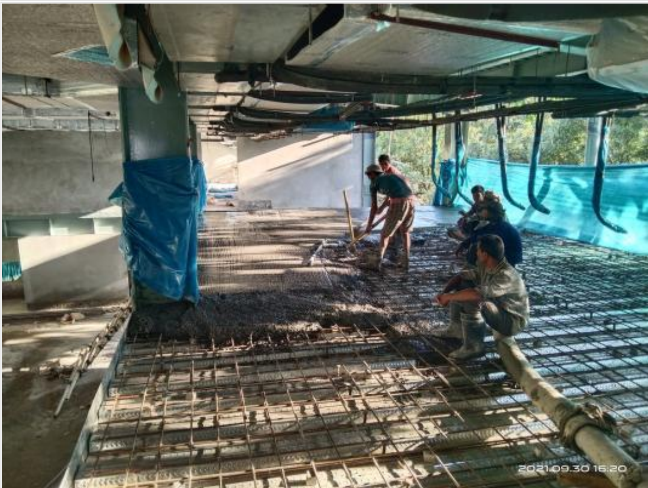
1F Mezzanine Slab Concreting on 30-09-21
