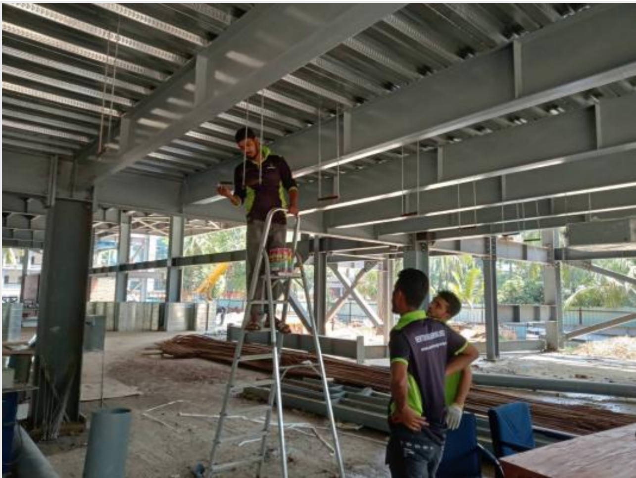
AC Duct Hanging on 22-05-21
