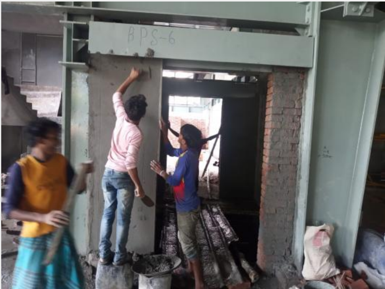
Lift door wall plaster on 22-09-21
