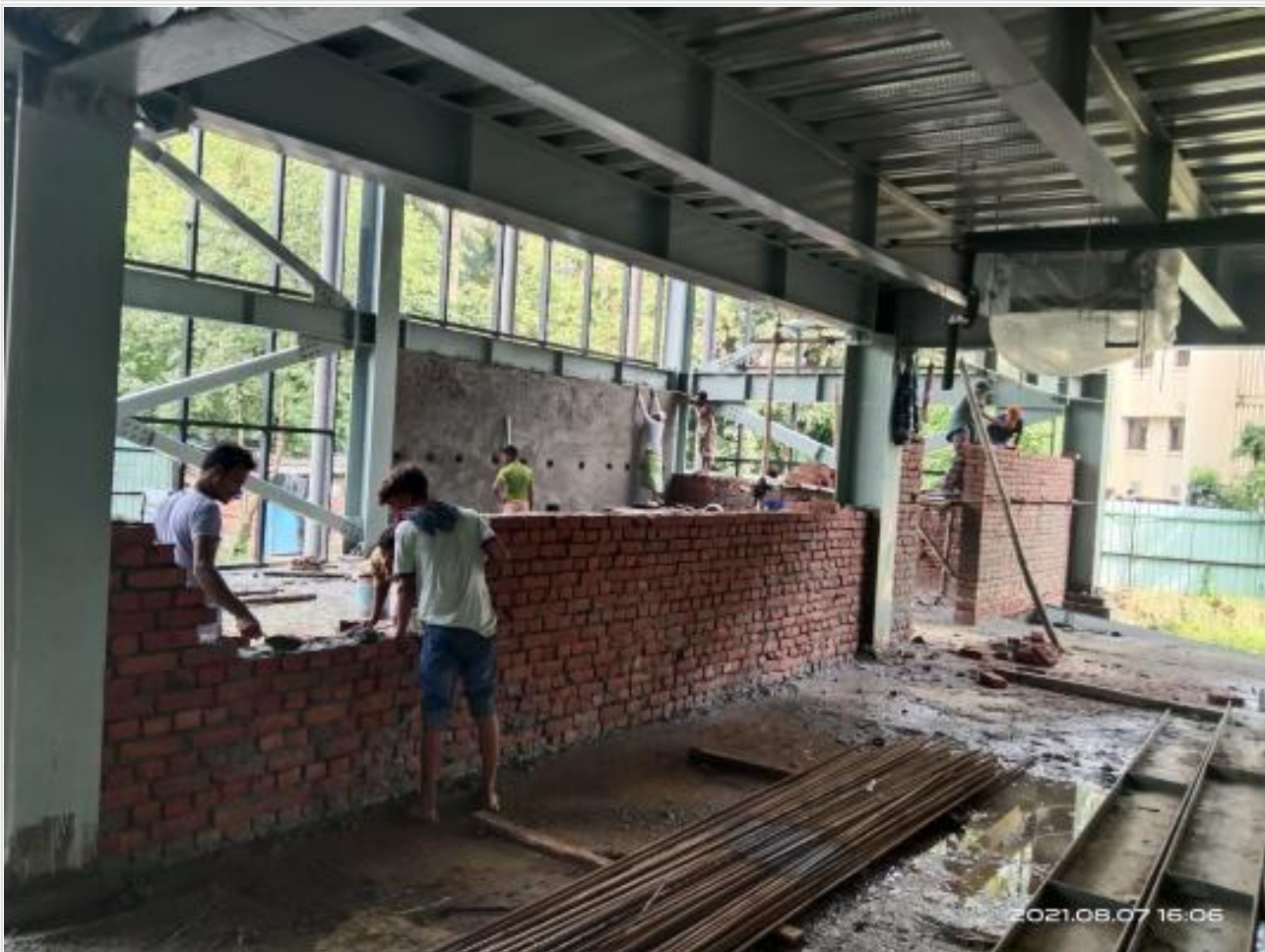
GF brick and plaster work on 07-08-21
