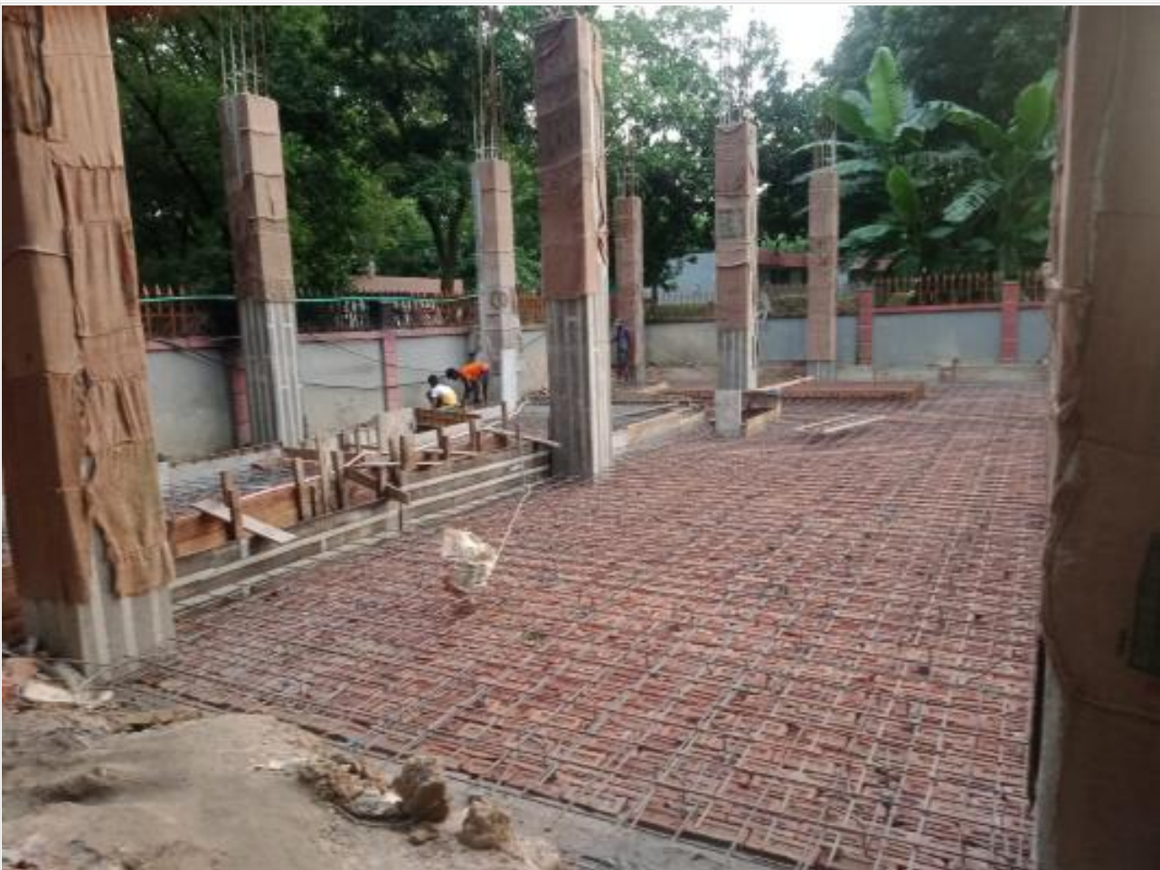
Generator room floor rod binding on 06-09-21
