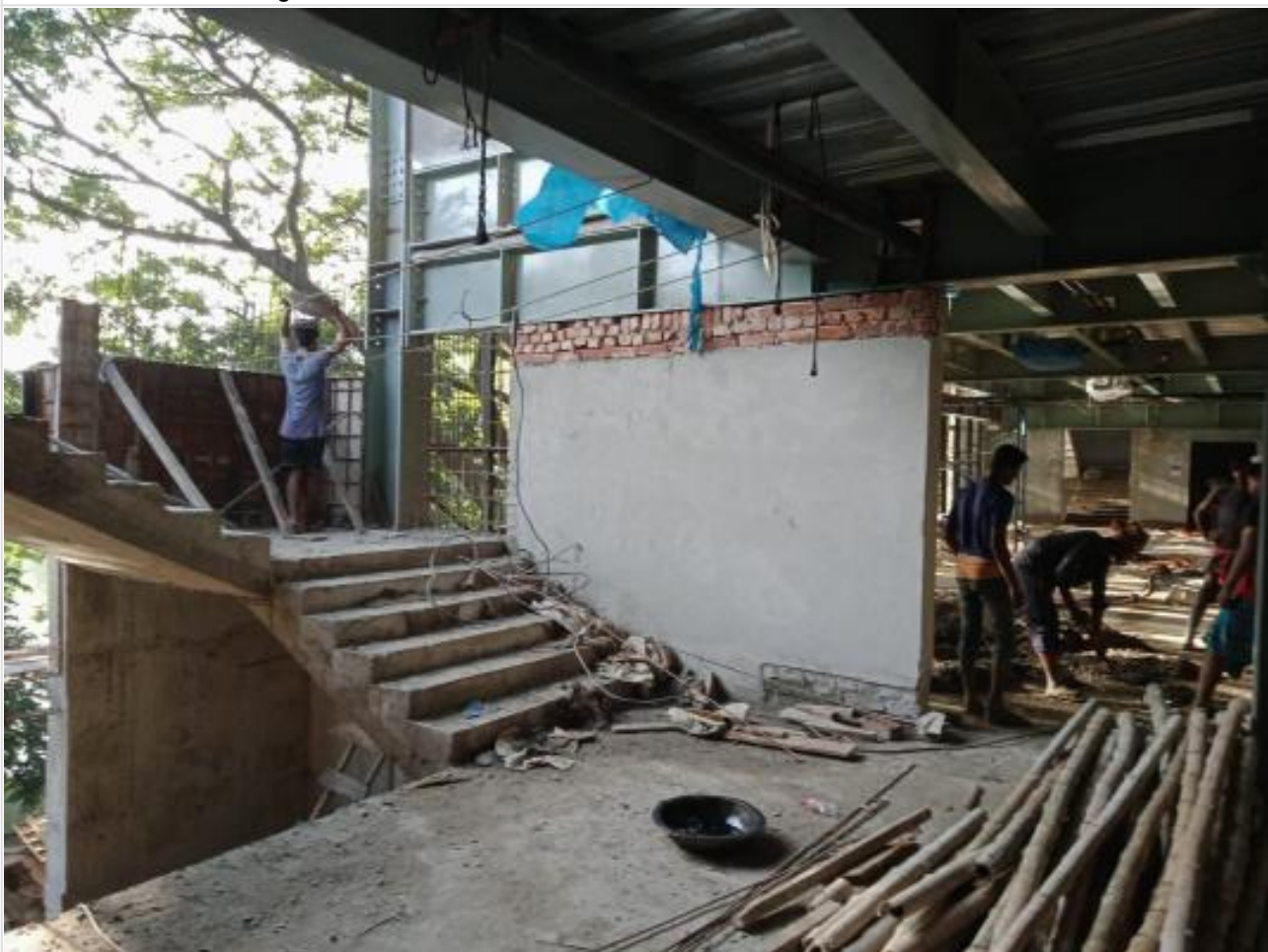
Stair RCC wall shuttering on 17-10-21
