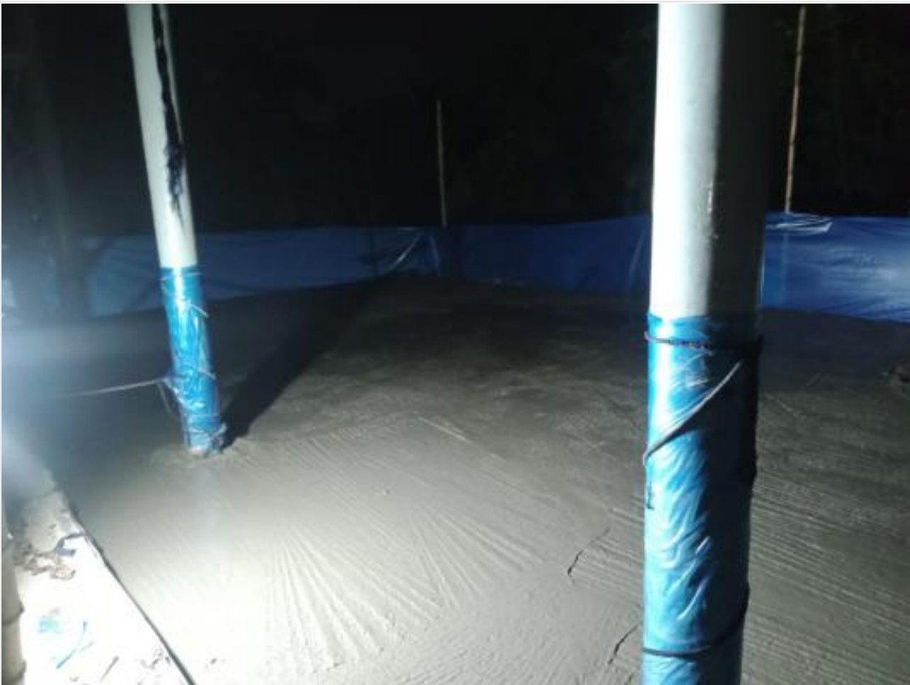
Porch Slab Concreting on 16-11-21
