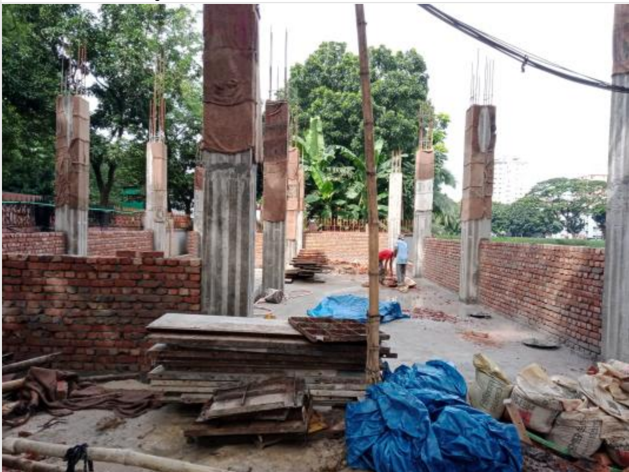
Generator room brick work on 10-09-21
