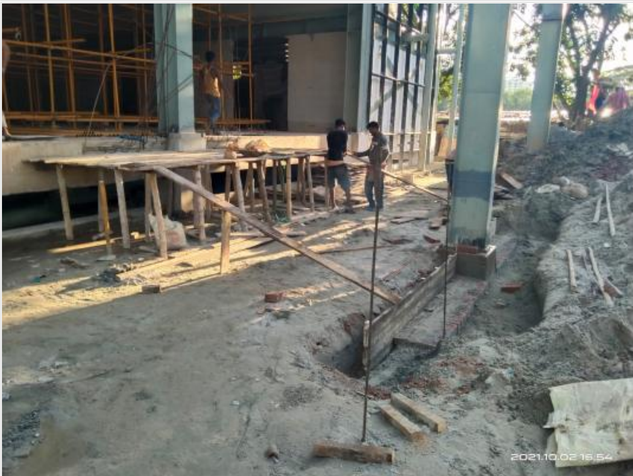
GF north entry stair work on 02-10-21
