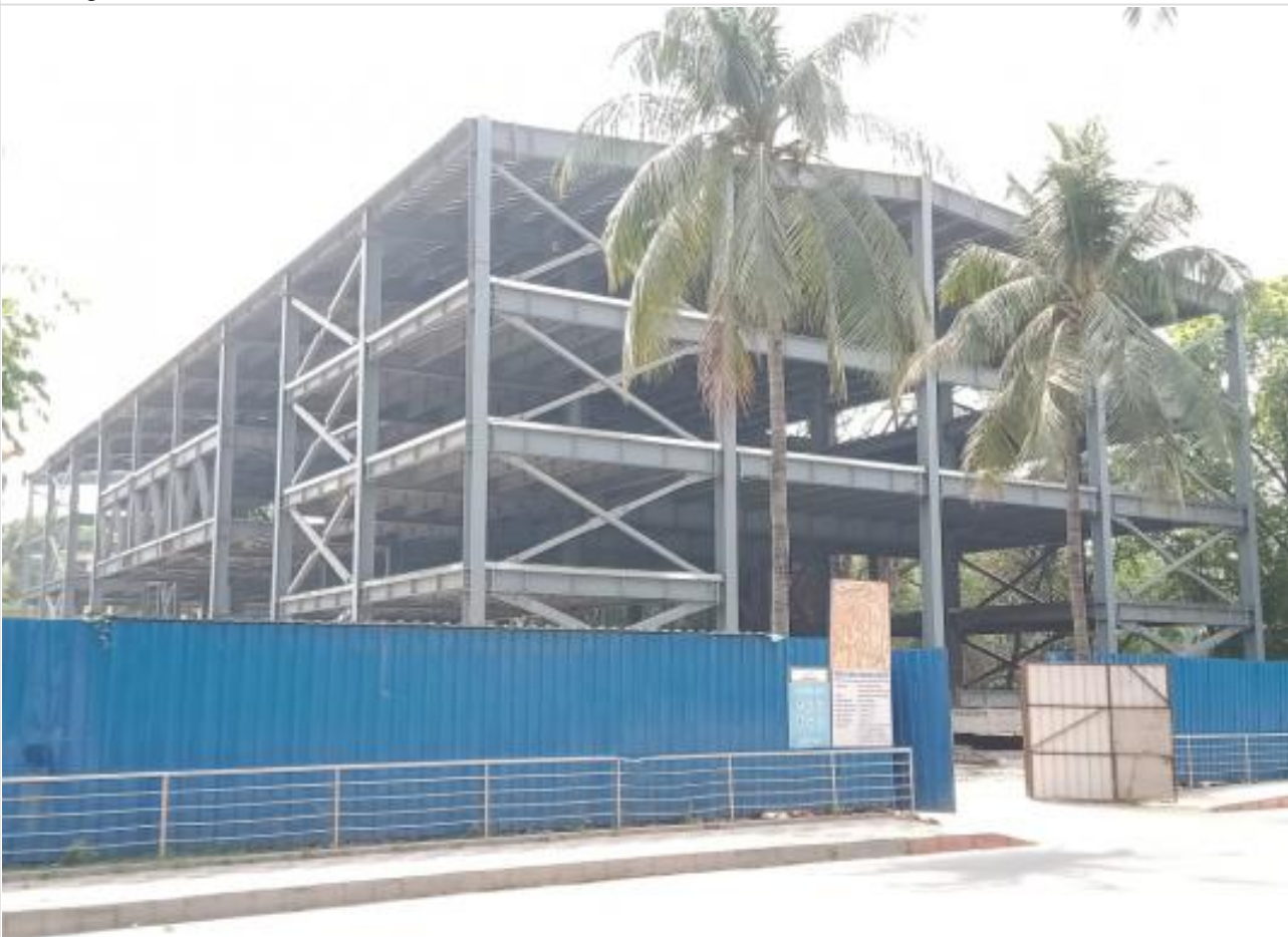
Decking Slab installation on 22-03-21
