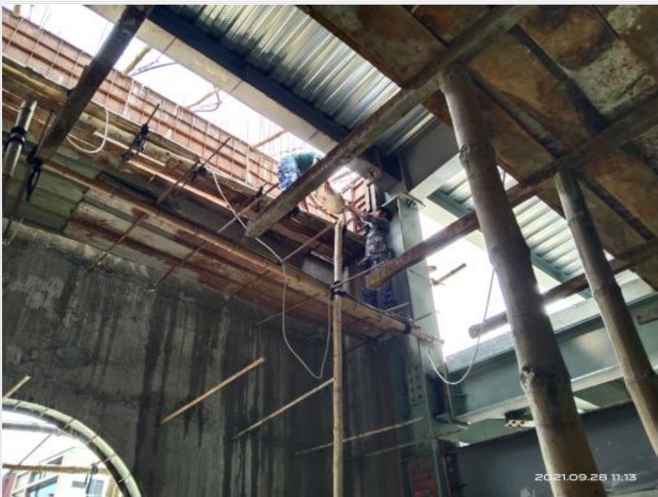
Stair wall casting on 28-09-21
