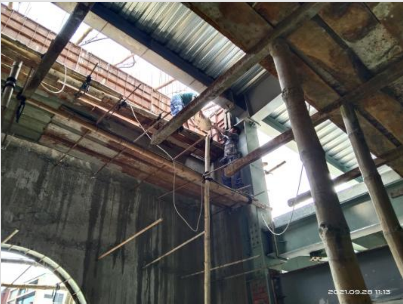
Stair wall casting on 28-09-21
