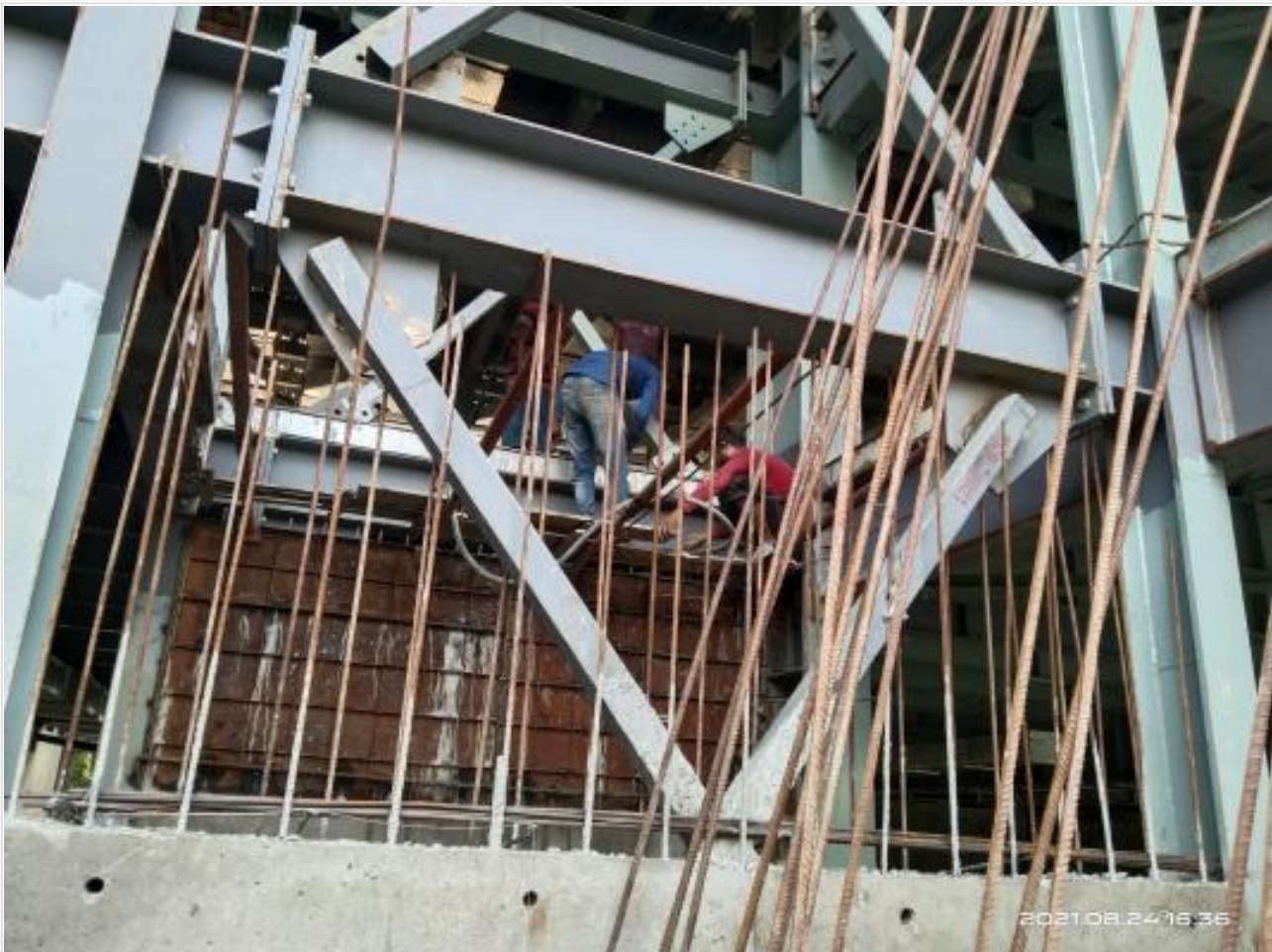
FFMezzanine stair casting on 24-08-21
