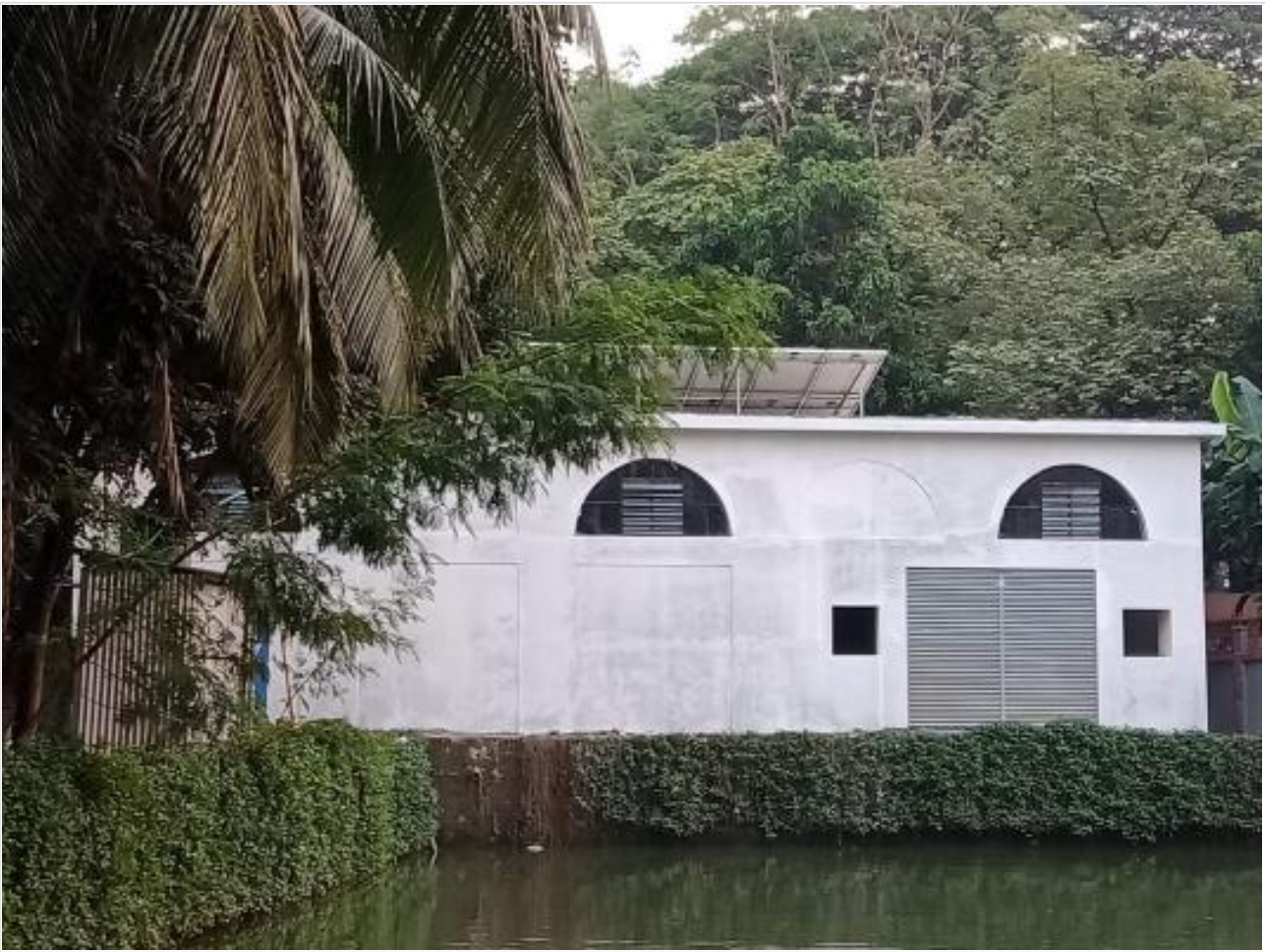
Generator room on 13-12-21
