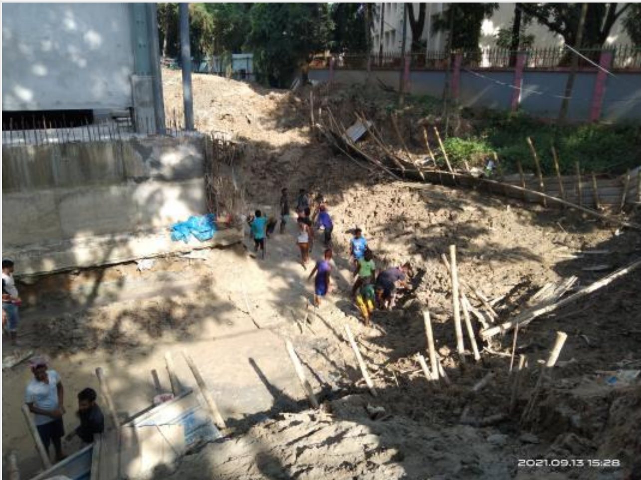
Fire tank clay remove on 13-09-21
