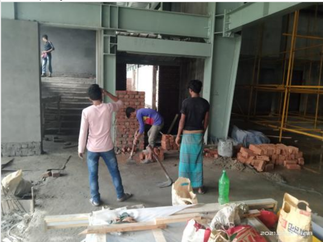
Lift front brick work as per opening on 21-09-21
