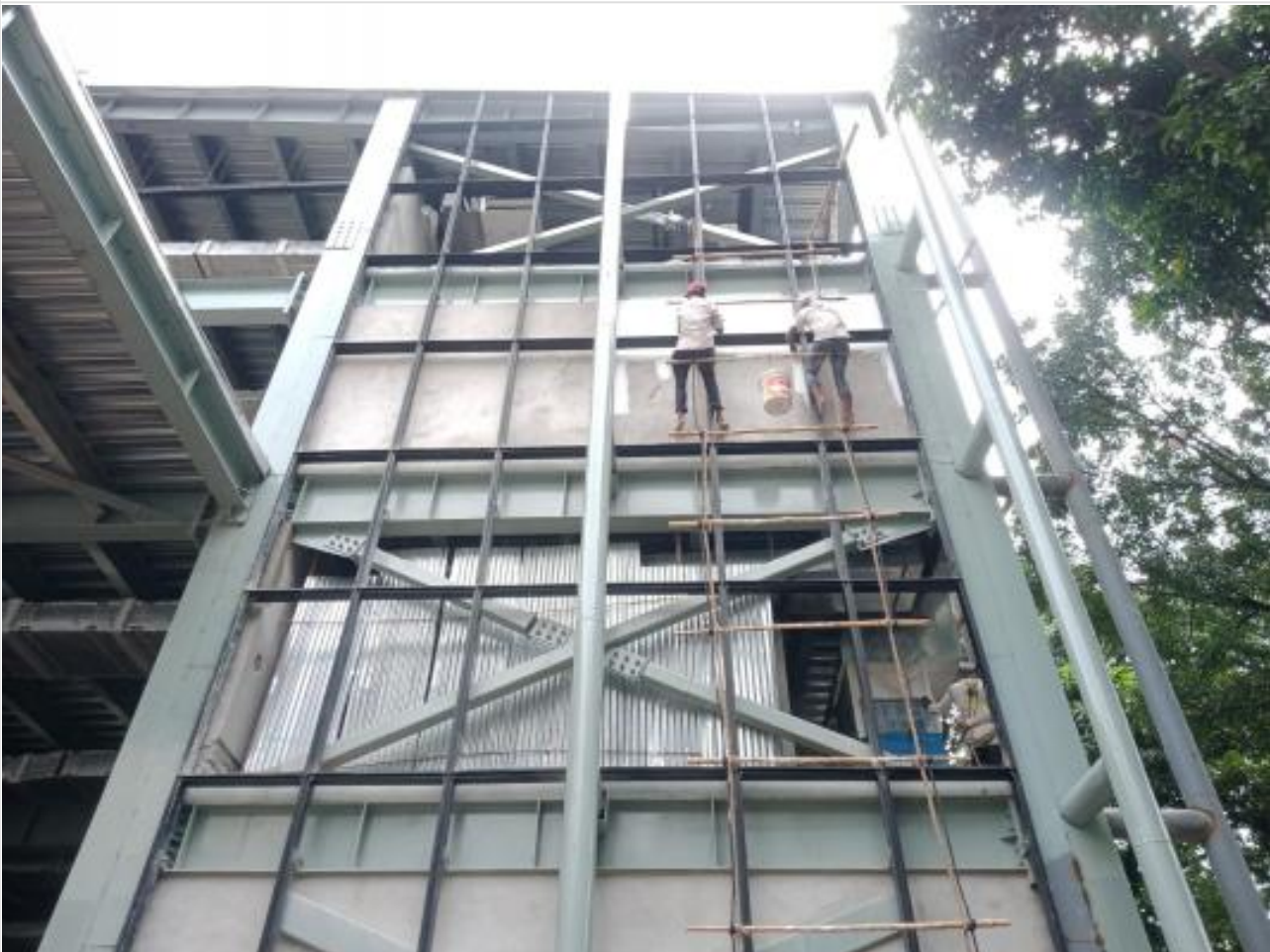
Outside painting work on 19-09-21
