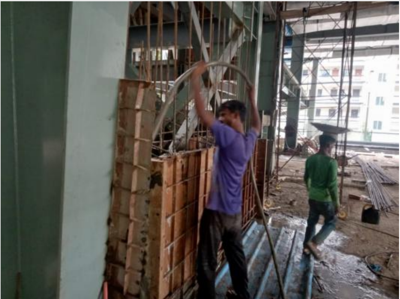
Ground Floor Lift Wall Concreting on 30-06-21
