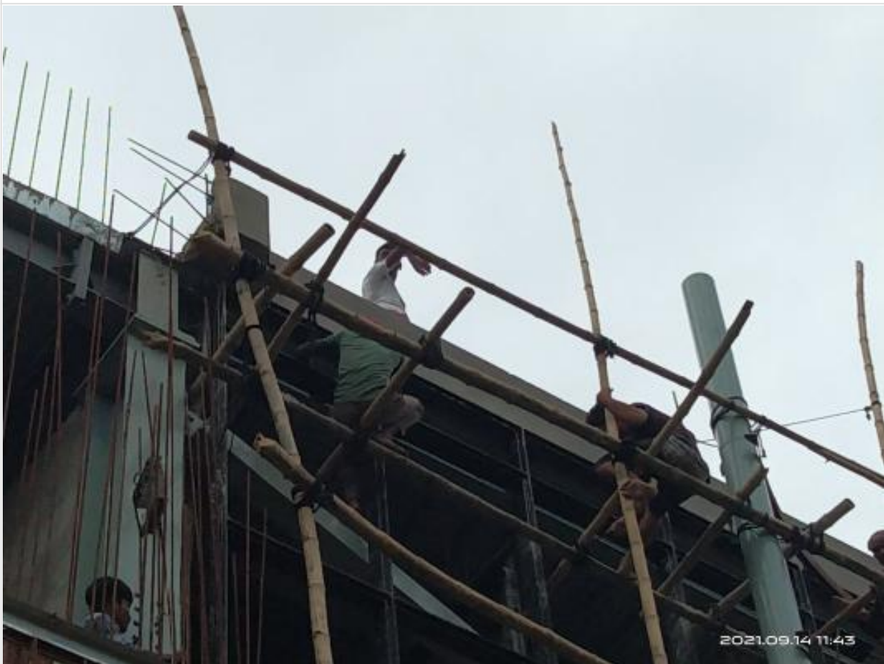
Gutter plaster work on 14-09-21
