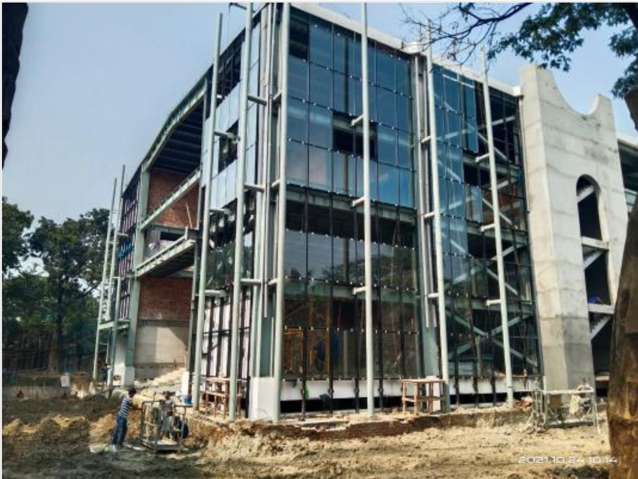
South East corner glass fitting on 24-10-21
