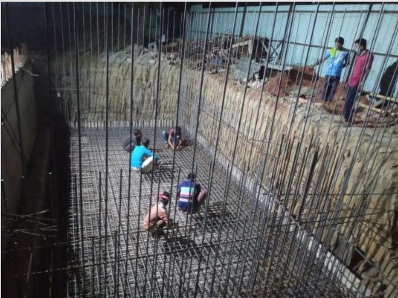
Domestic Water Tank Re-bar work on 01-05-21
