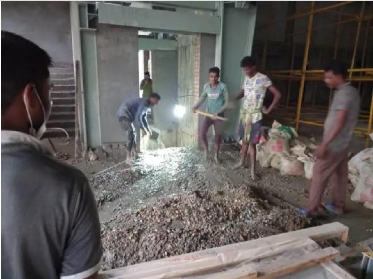
Stair wall casting on 25-09-21
