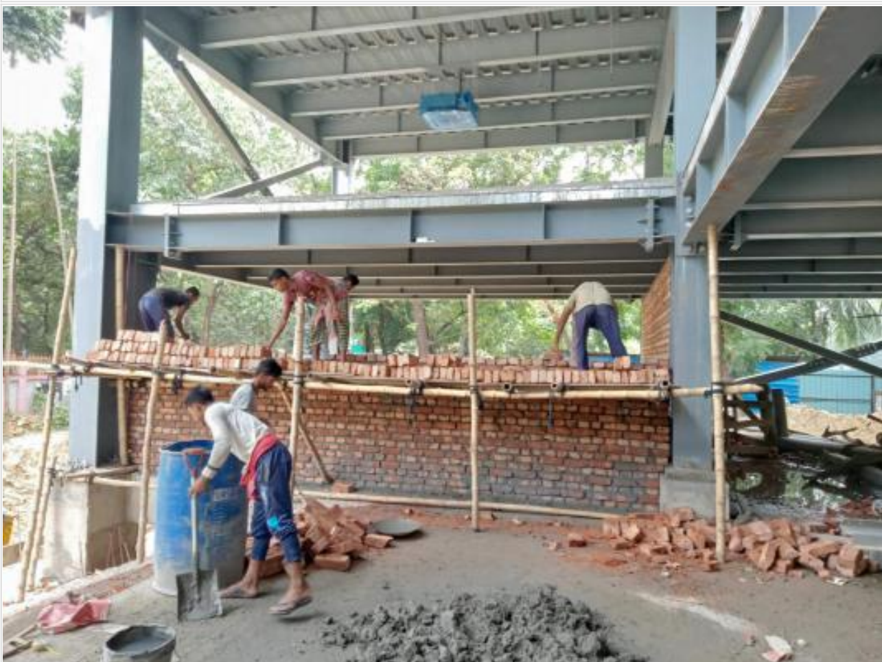
Ground Floor Brick Work on 25-05-21
