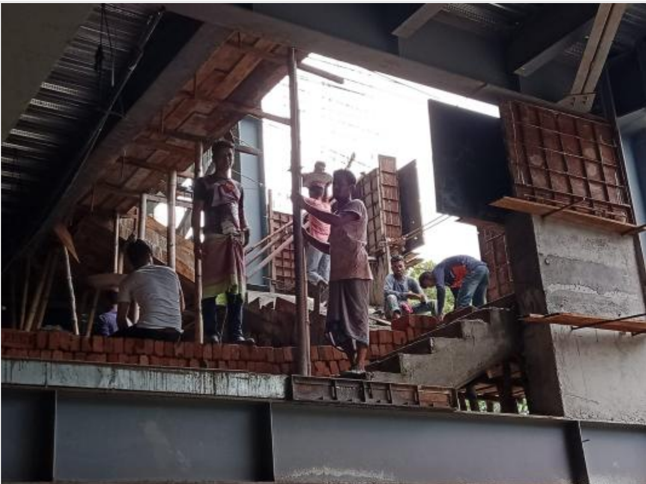
GF Mazzanine stair wall casting on 04-08-21
