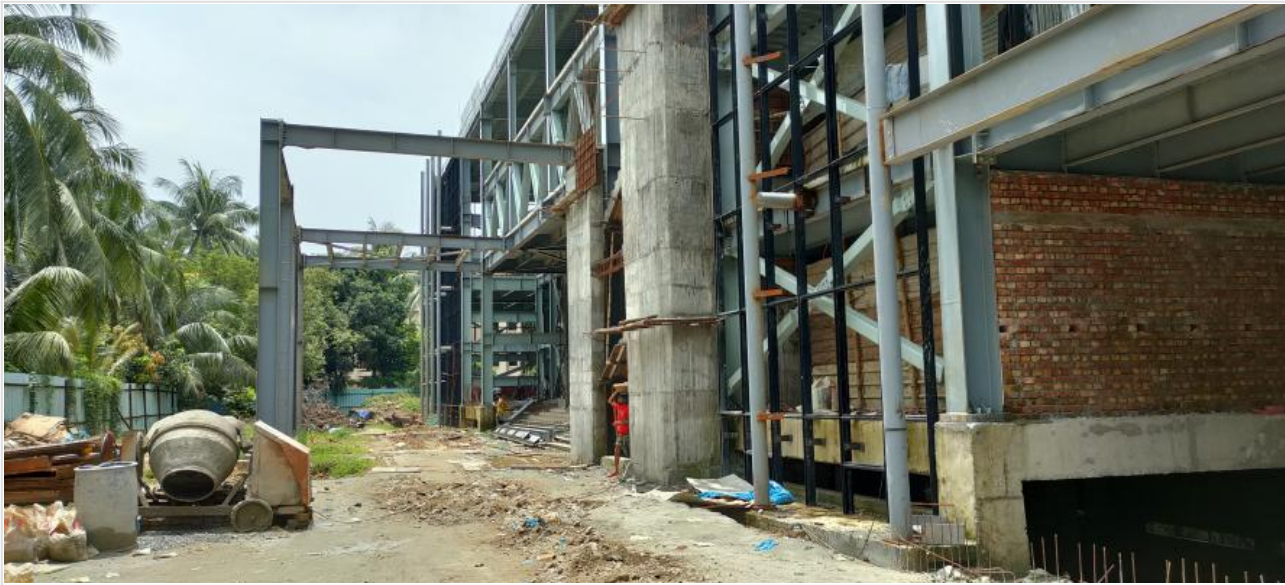
Steel Canopy Installing on 06-08-21
