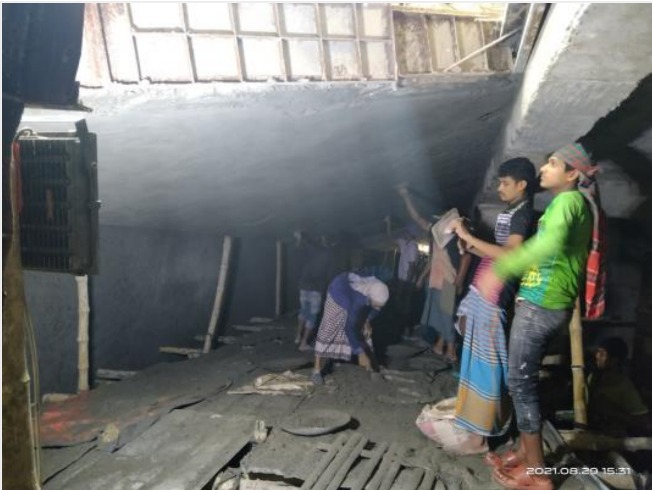
Basement ceiling plaster on 29-08-21
