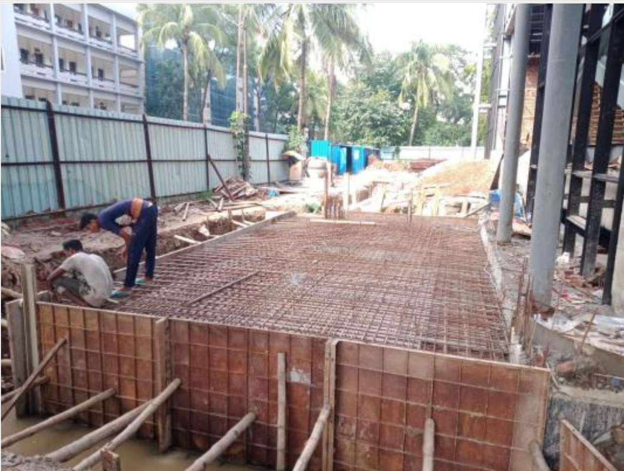
Domestic Water Tank Slab Re-barwork on 23-06-21
