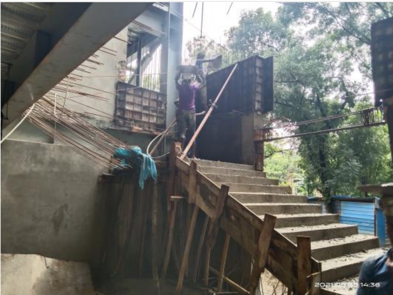
Stair wall casting (stair-4) on 09-09-21
