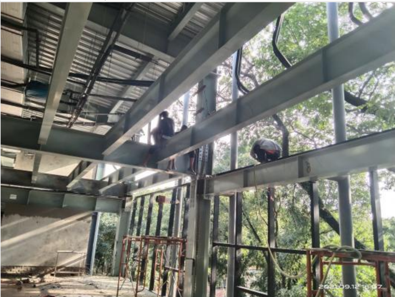
Retrofitting work at 1st floor mezzanine on 12-09-21
