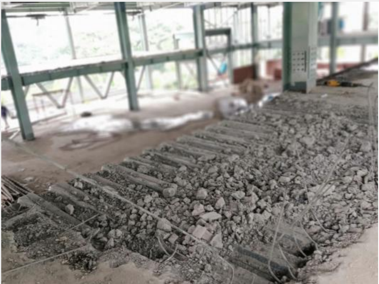
FF Mezzanine floor dismantling work on 18-08-21
