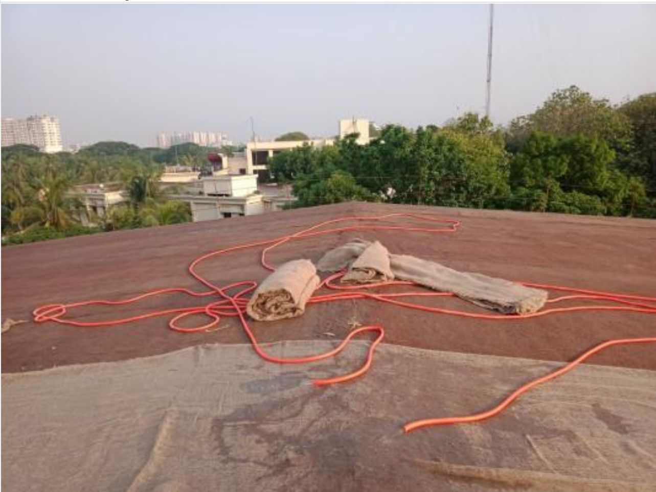
Hessian Cloth Covering after Concreting on 06-05-21
