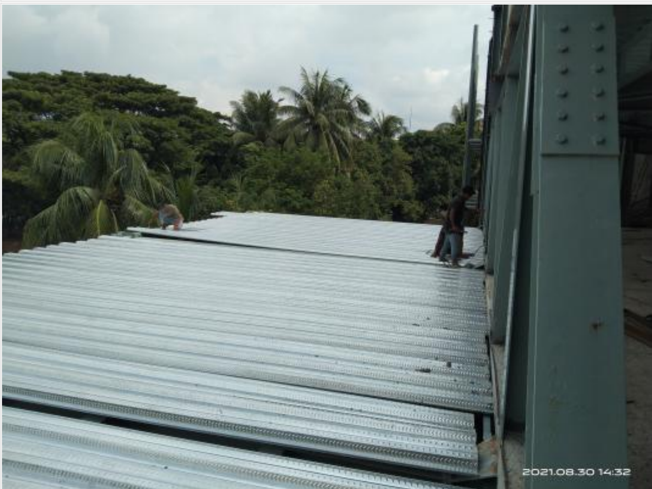
East Canopy decking sheet shitting on 30-08-21
