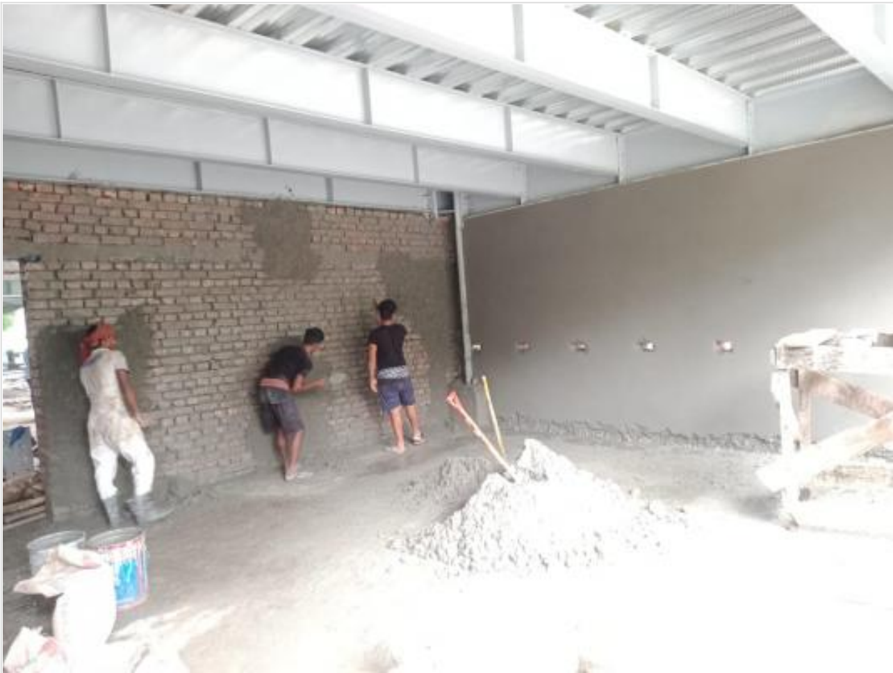
Ground Floor-Plastering on 30-06-21
