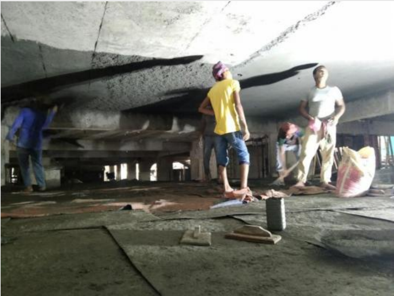
Basement Ceiling Plastering on 09-06-21
