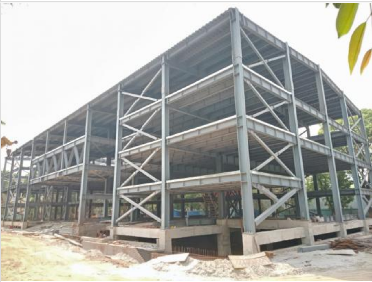
Decking Slab installation on 05-04-21
