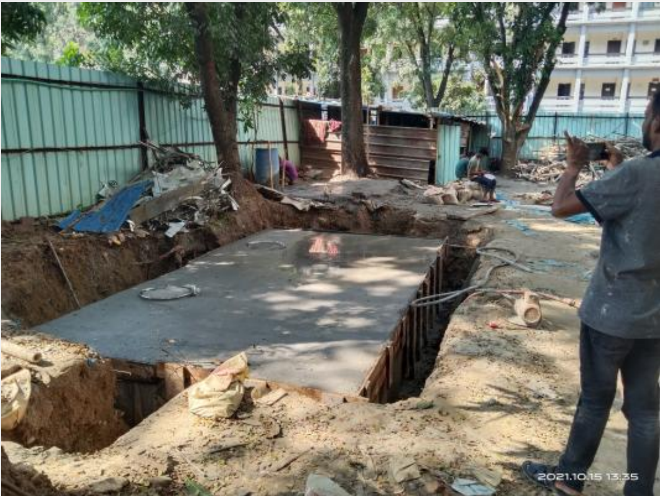
Septic tank top slab casting on 15-10-21
