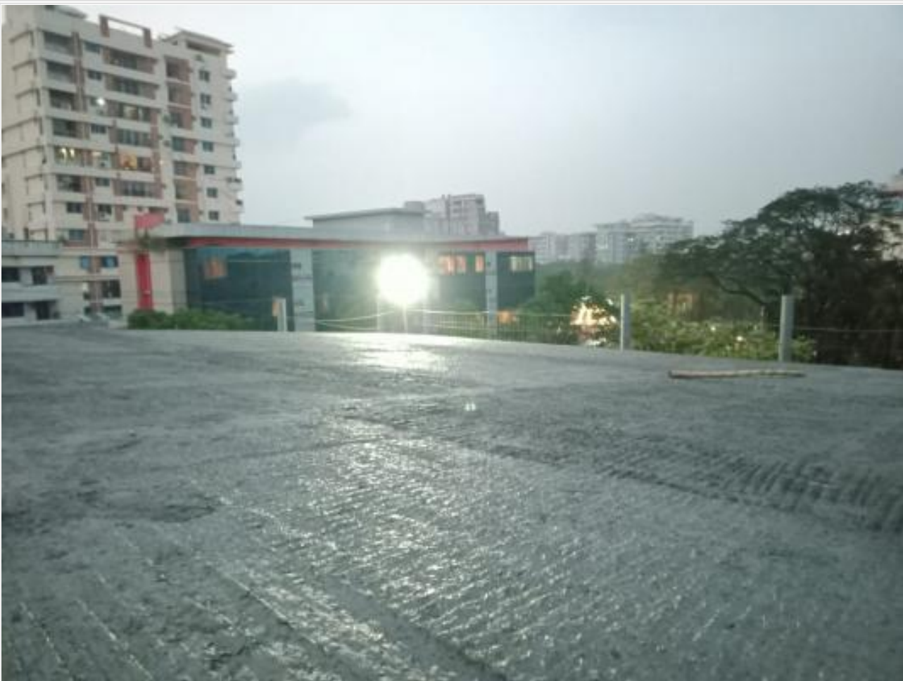
Roof Slab Concreting Completed on 07-05-21
