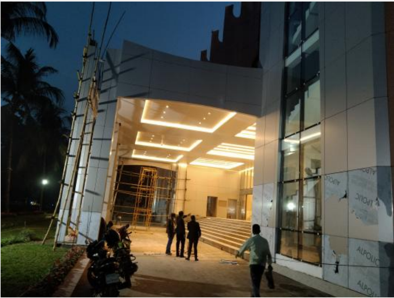
Interior works on 16-12-21
