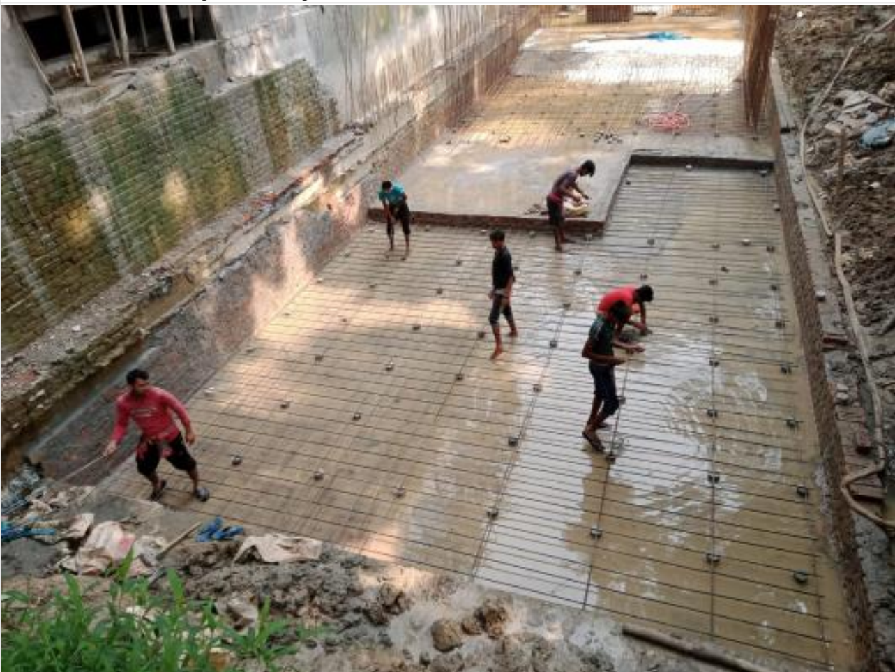
Fire tank base rod binding on 12-10-21
