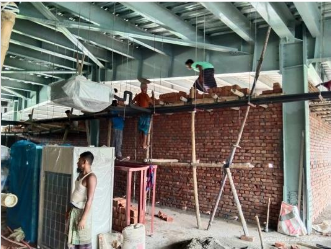
FFM brick wall on 25-08-21
