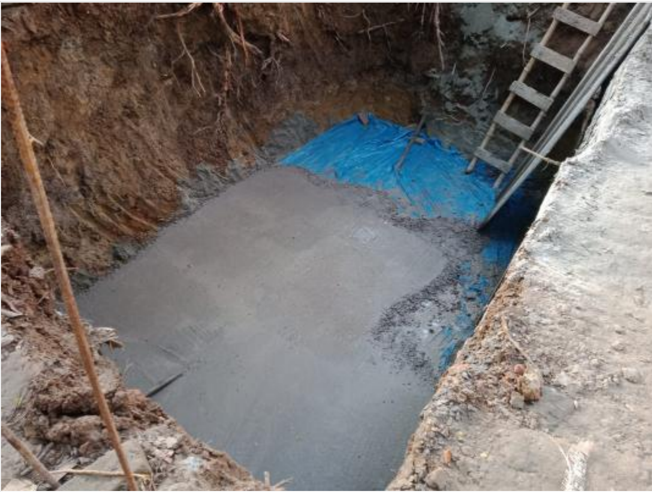
Septic tank cc work on 15-09-21
