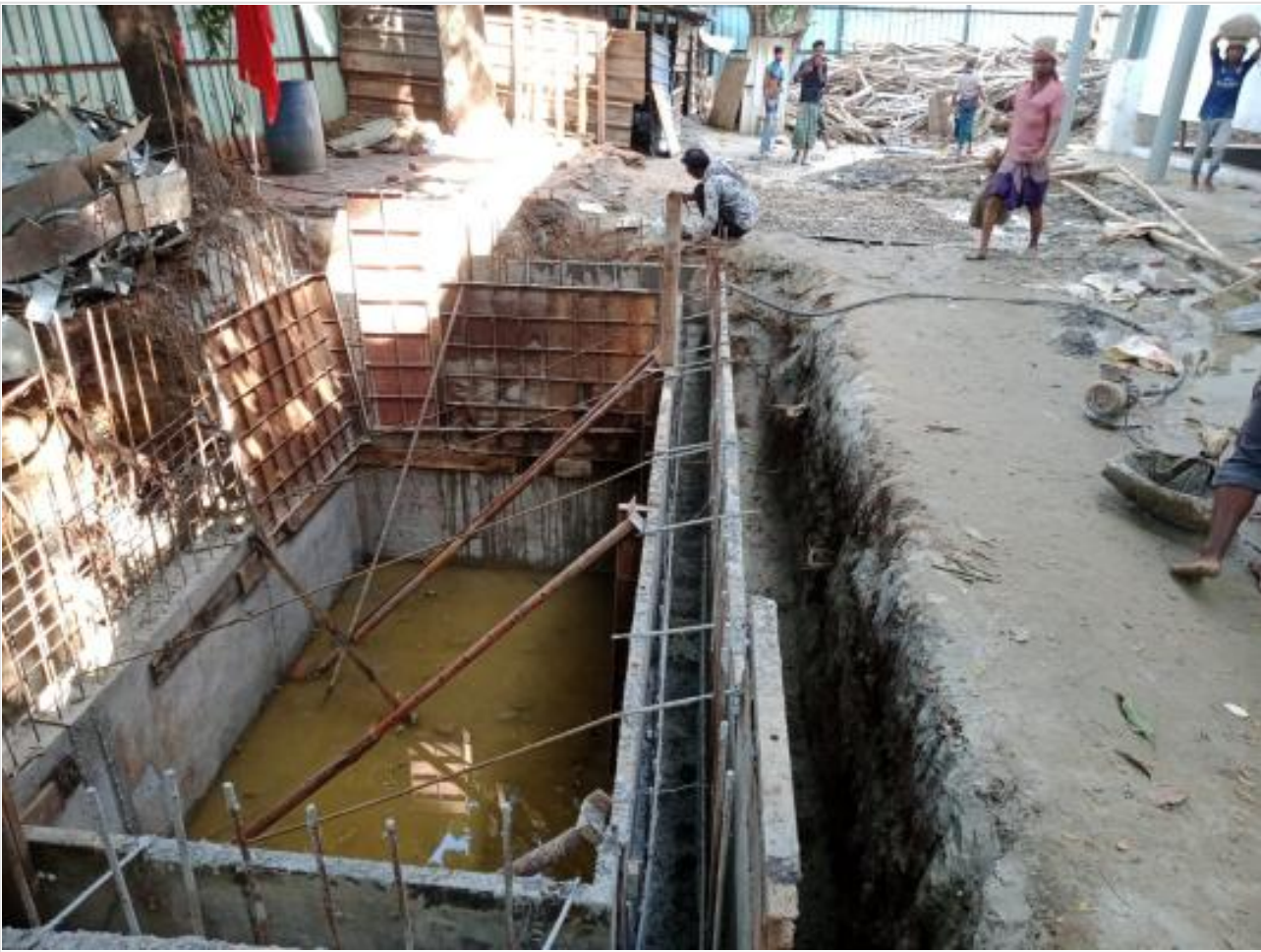
Septic tank wall shuttering on 01-10-21
