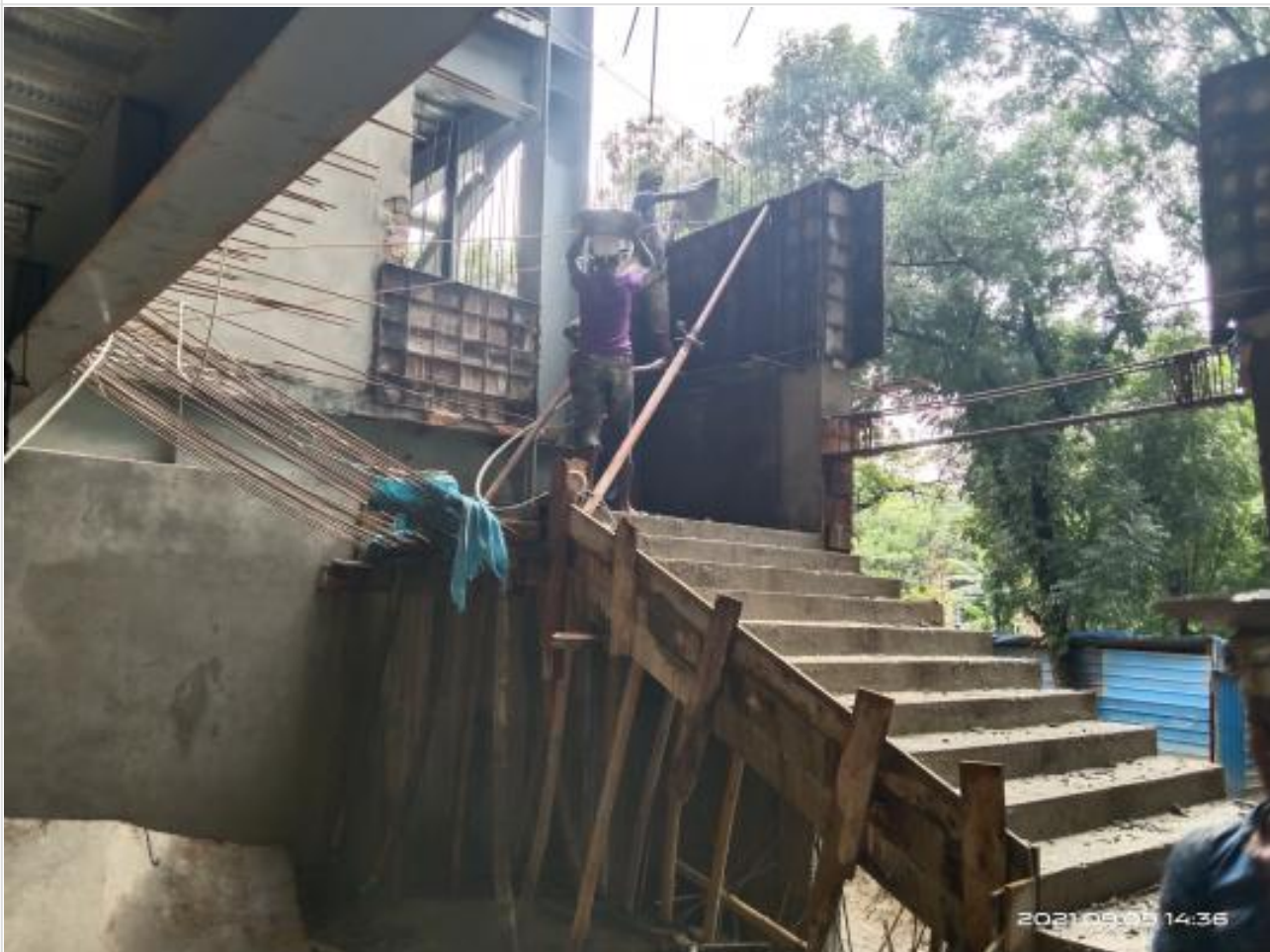
Stair wall casting (stair-4) on 09-09-21
