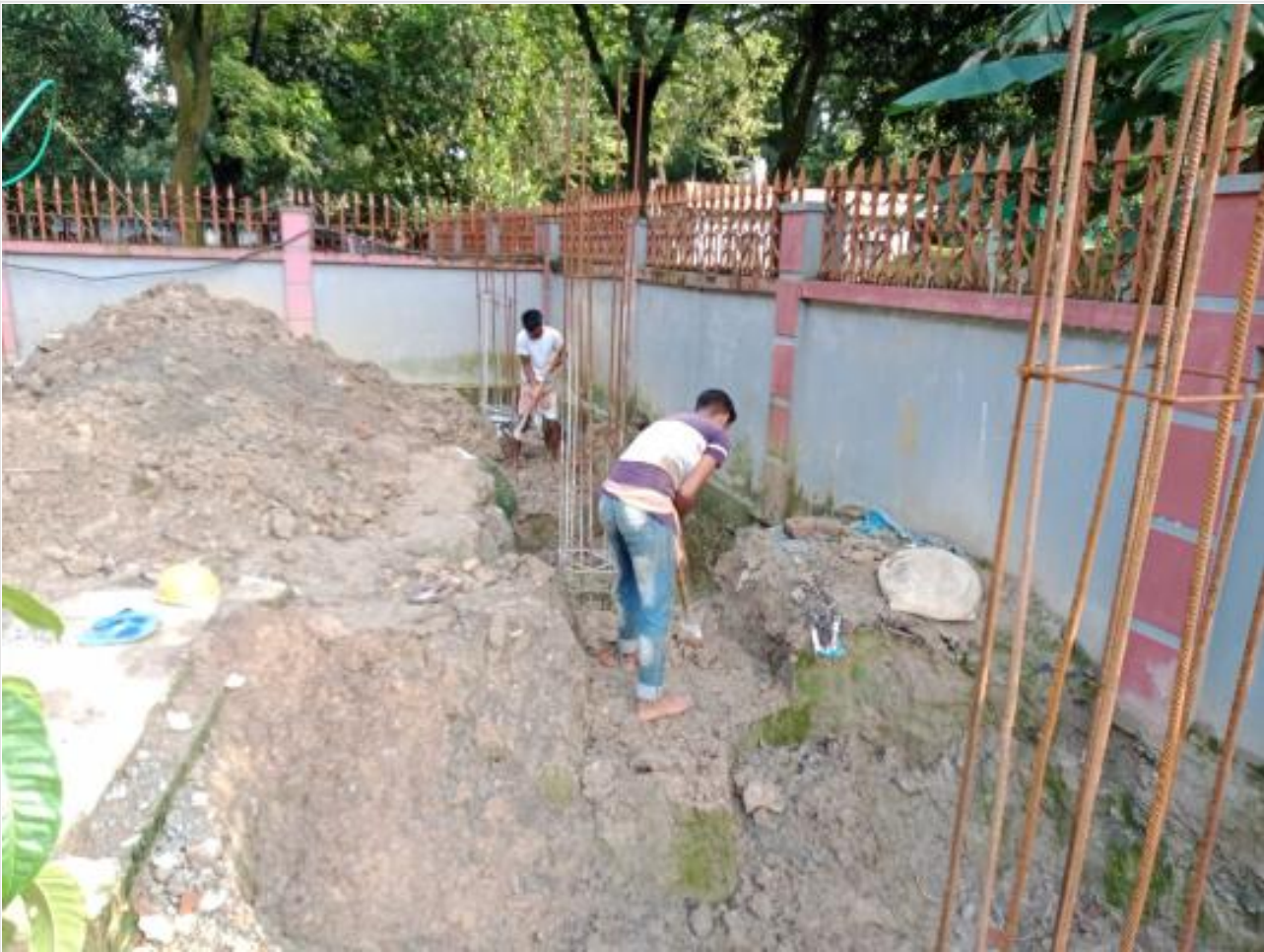
Sub-station grade beam earth cutting on 01-08-21
