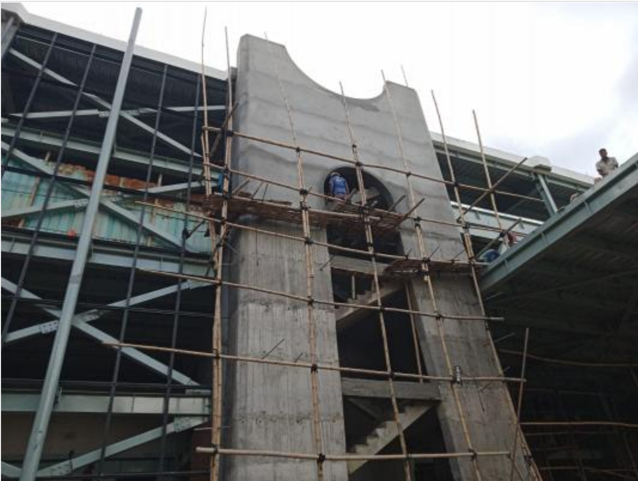
Outside stair plaster on 18-10-21
