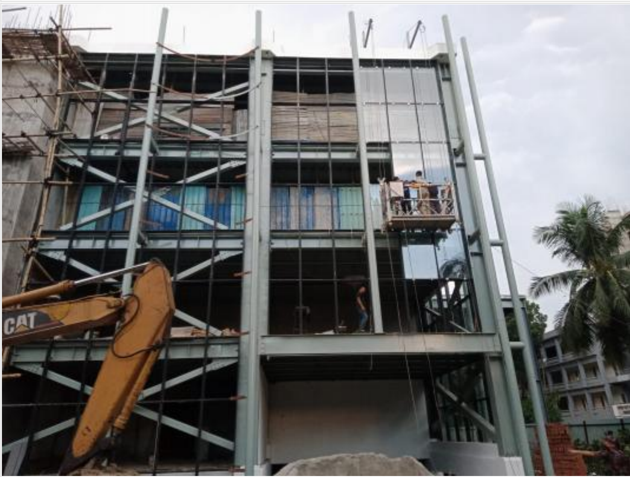
Glass fitting work on 27-09-21
