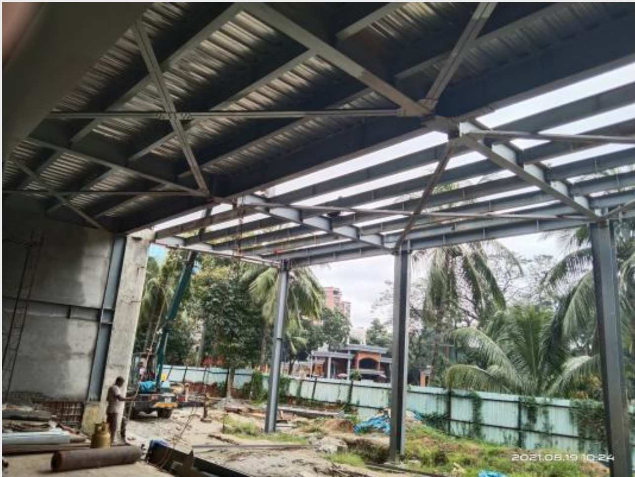
East steel canopy on 19-08-21
