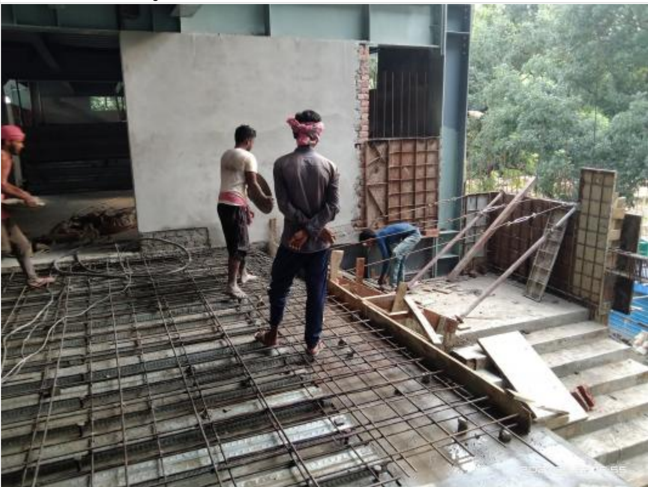
GF Mezzanine stair casting (4-no) on 23-09-21
