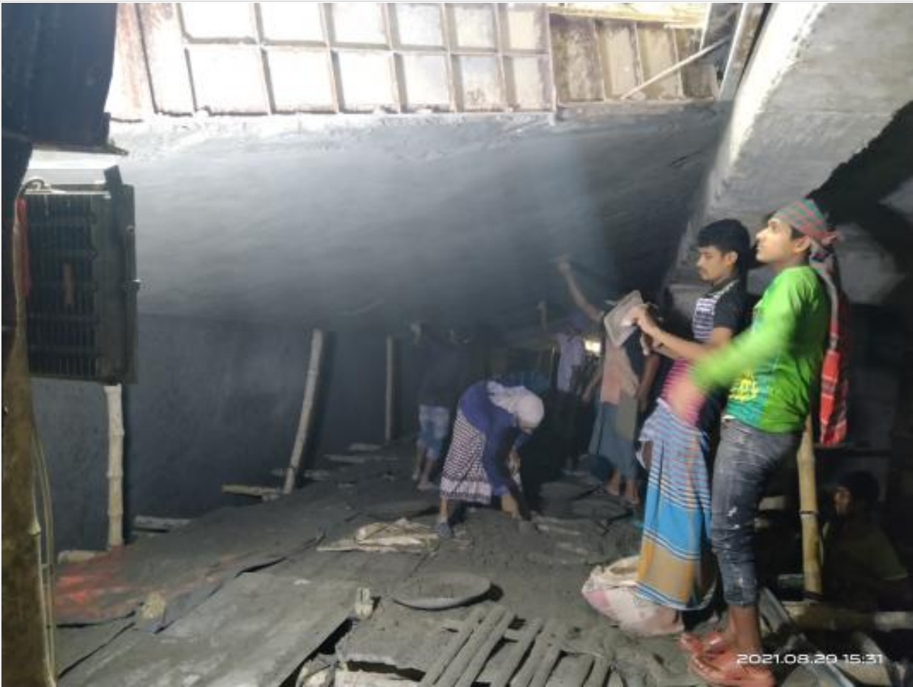
Basement ceiling plaster on 29-08-21
