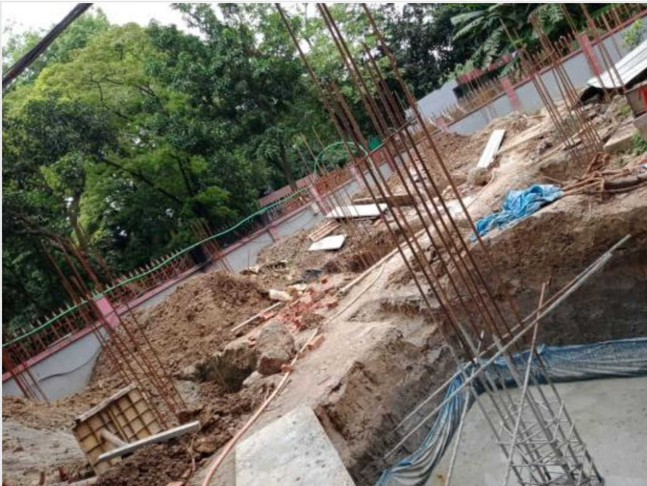
Substation Footing Concreting on 18-07-21
