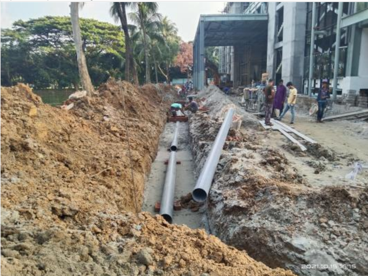
Under ground uPVC pipe line work on 15-10-21
