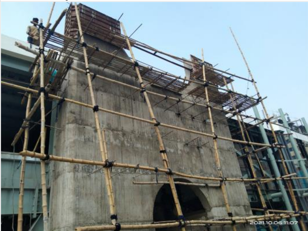
Stair wall casting of stair no. 02 on 06-10-21
