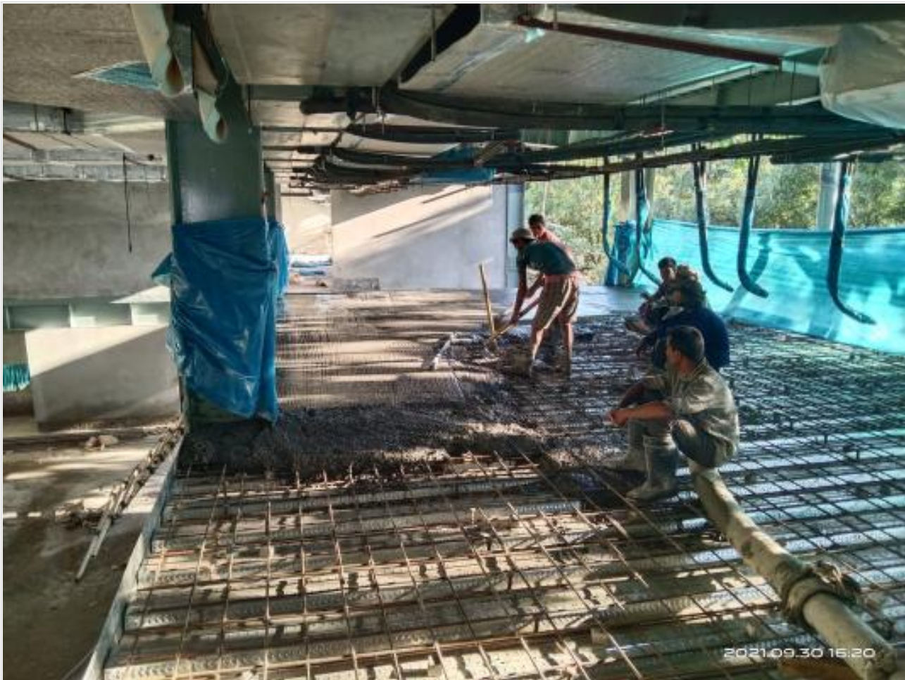
1F Mezzanine Slab Concreting on 30-09-21
