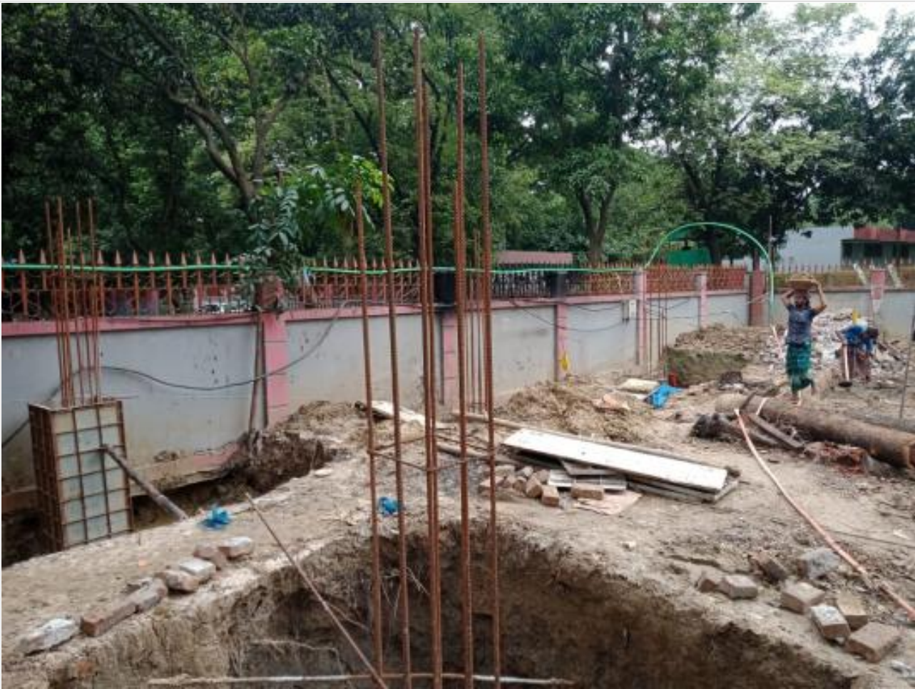
Substation-Generator Room-Excavation on 27-06-21
