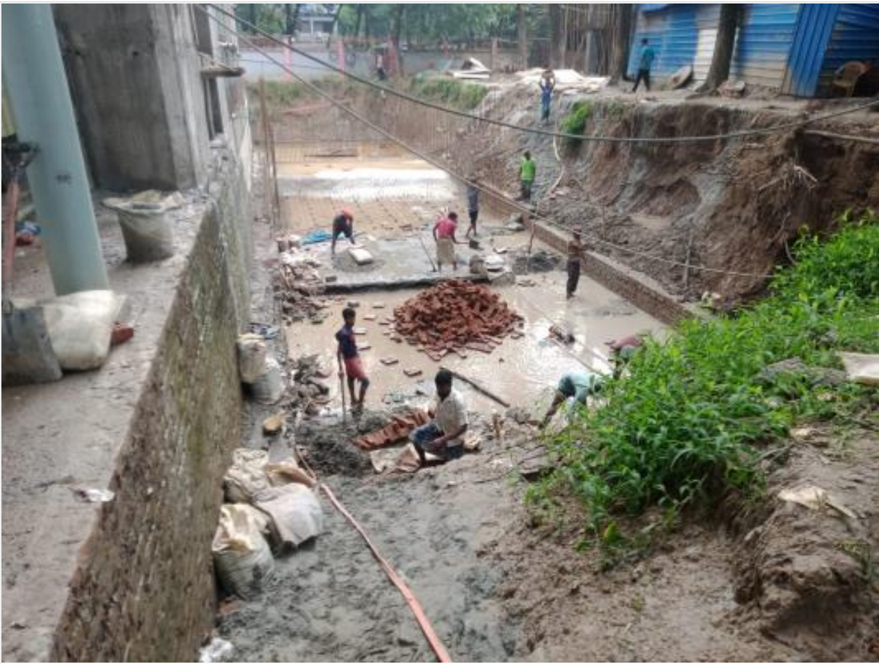
Fire Tank clay protection wall making on 08-10-21
