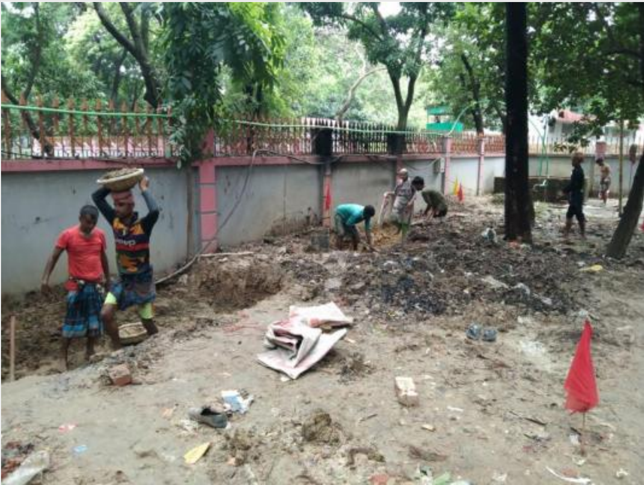
Substation n Generator Base excavation on 07-06-21
