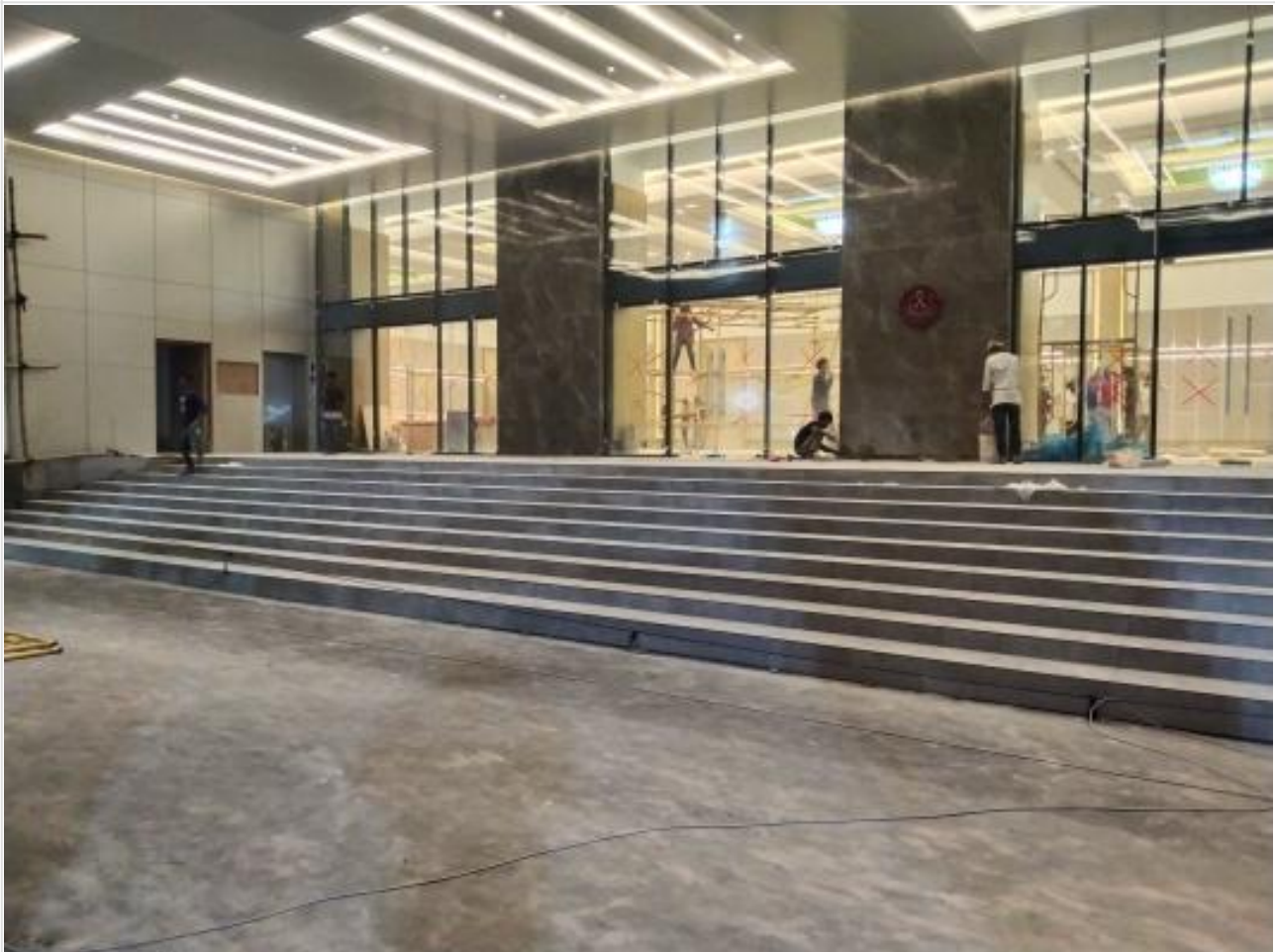
East entry on 14-12-21
