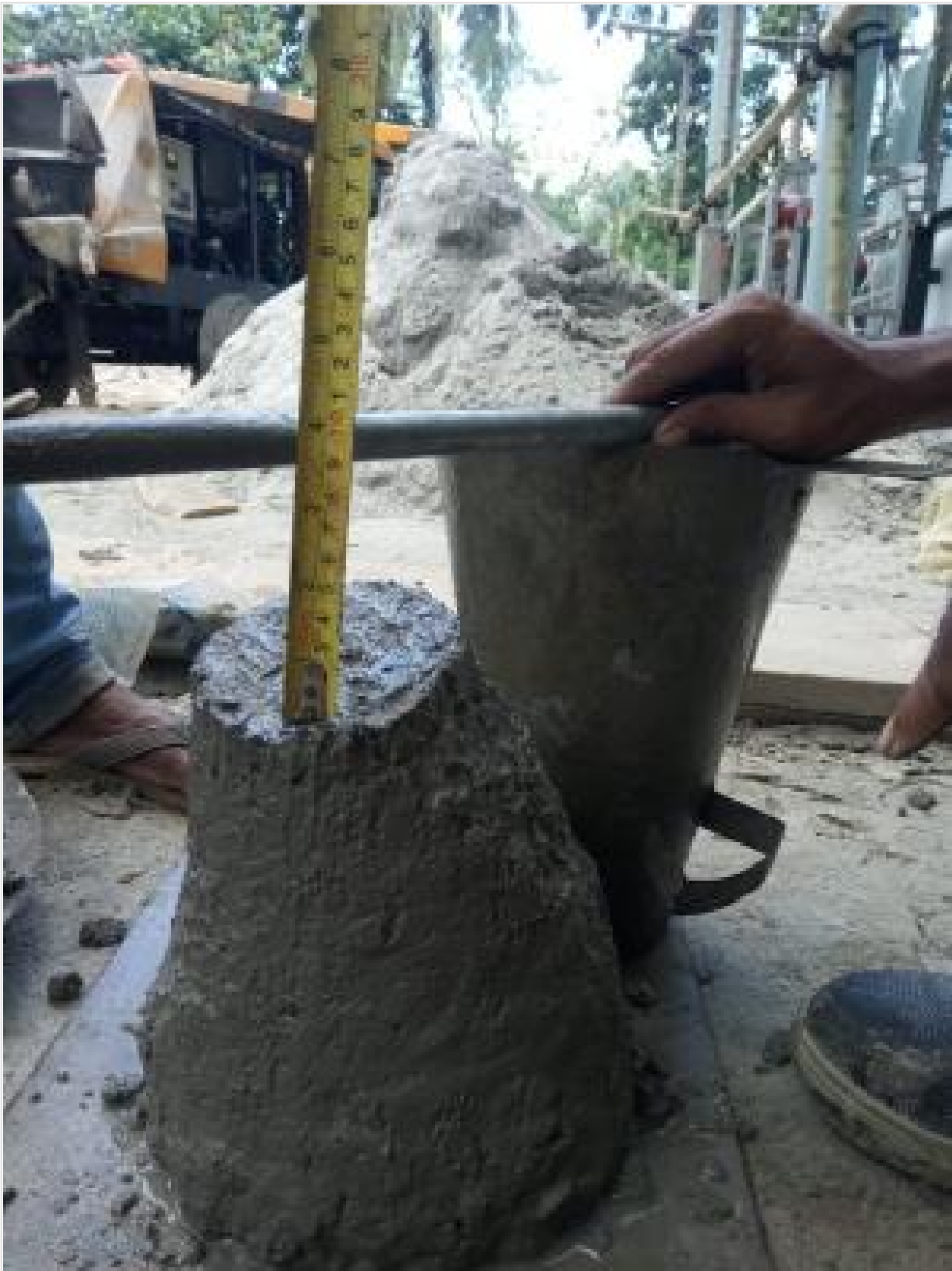
Generator floor casting Slump Test on 08-09-21
