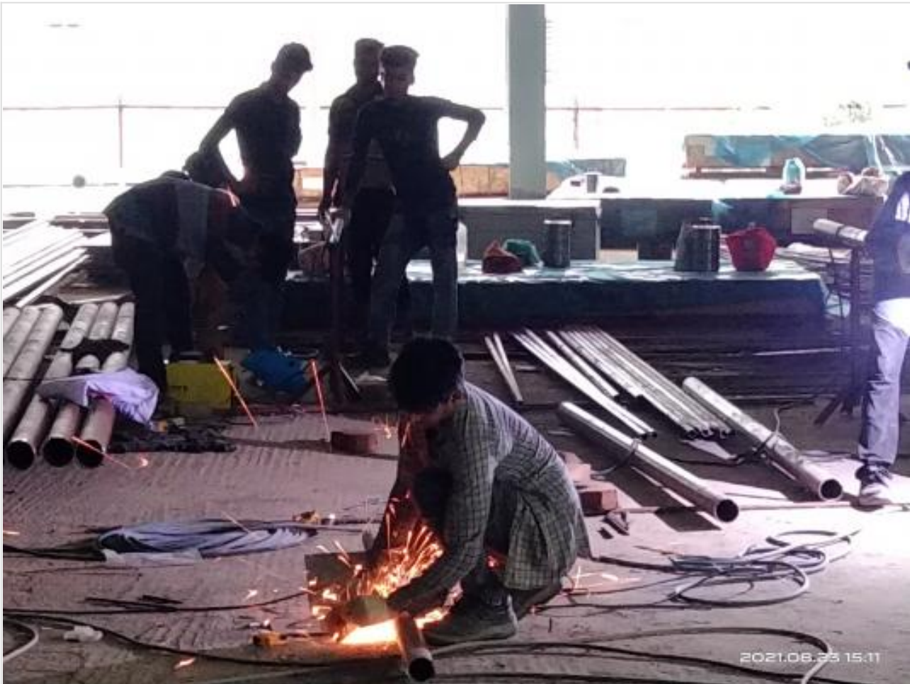
Piping work for fire on 23-08-21
