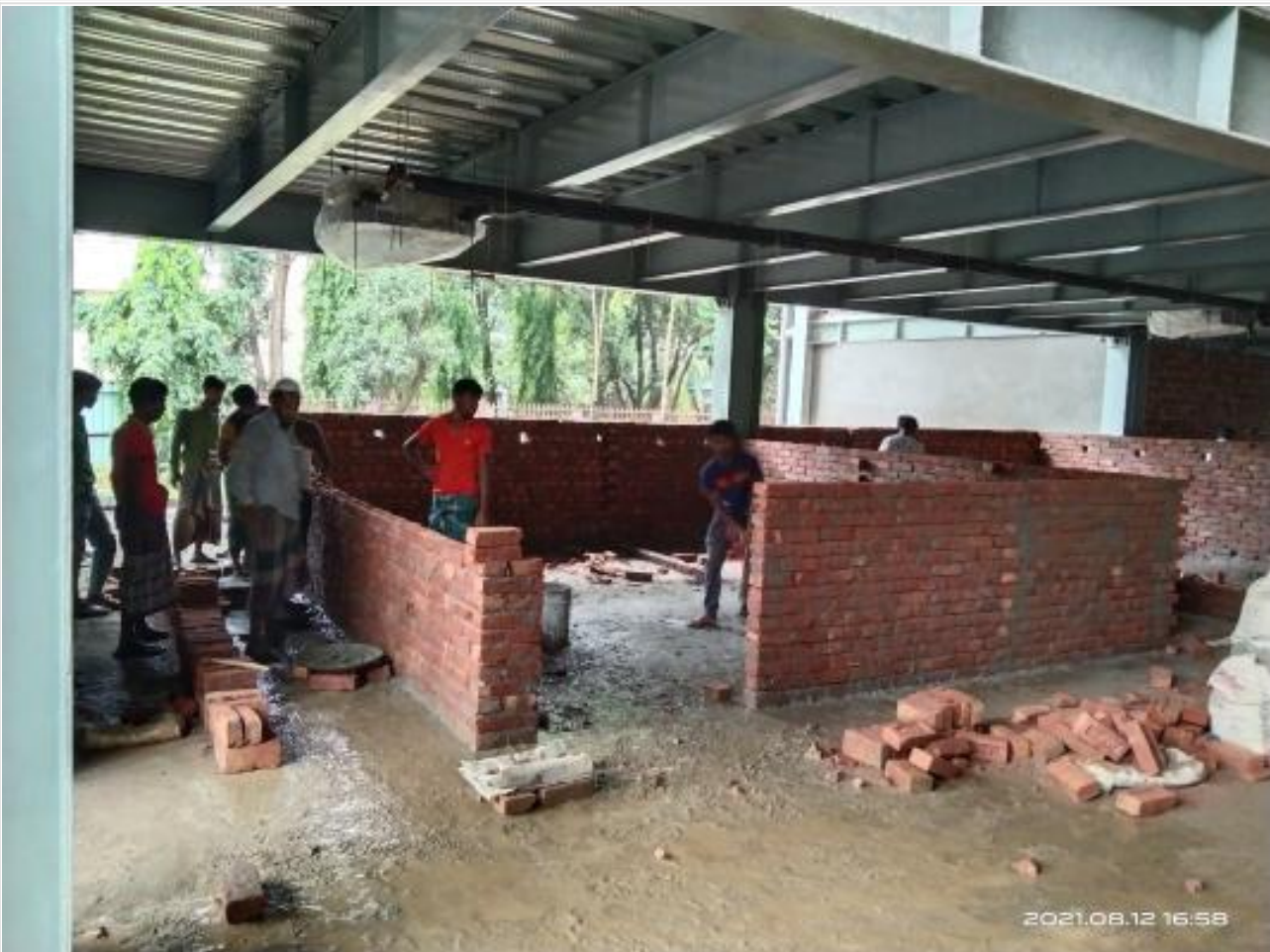
GF Brick work on 12-08-21
