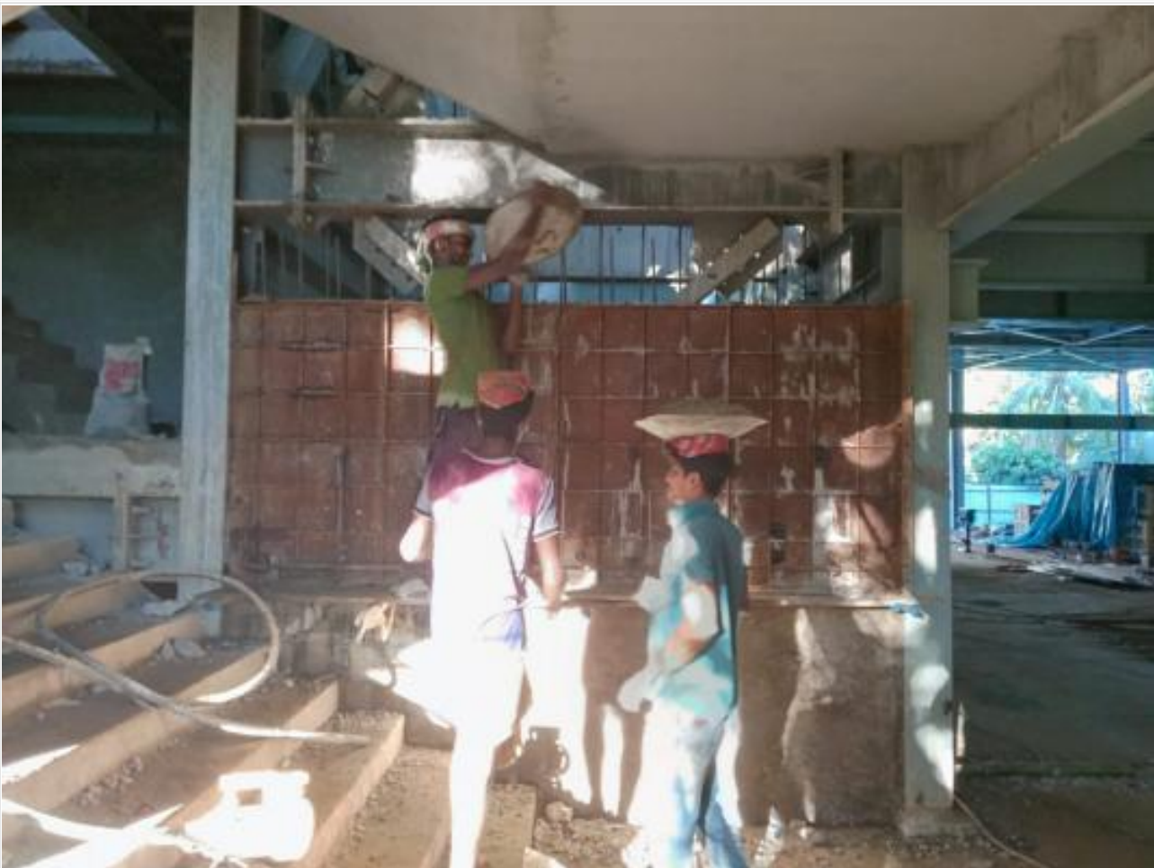
GF Lift wall Casting on 31-08-21
