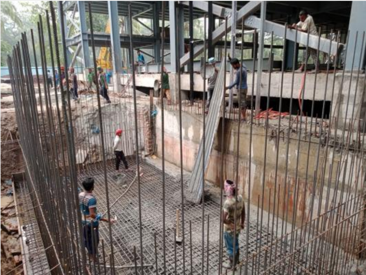
Domestic Water Tank Base concreting on 03-05-21
