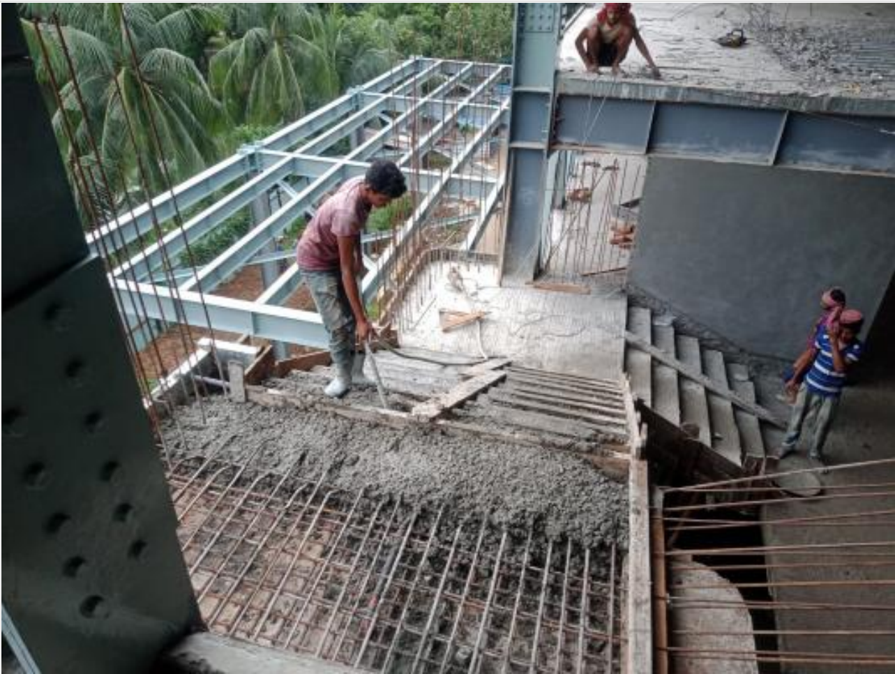
FF Mezzanine stair casting on 21-08-21
