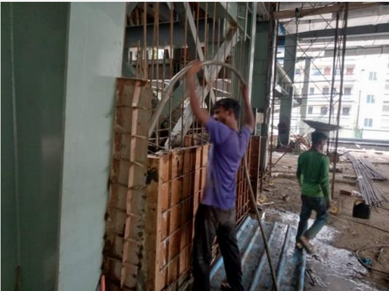
Ground Floor Lift Wall Concreting on 30-06-21
