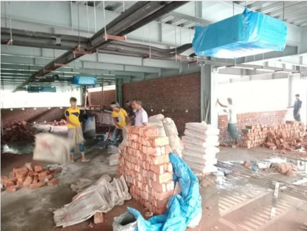
GF merzzanine brick work on 03-08-21
