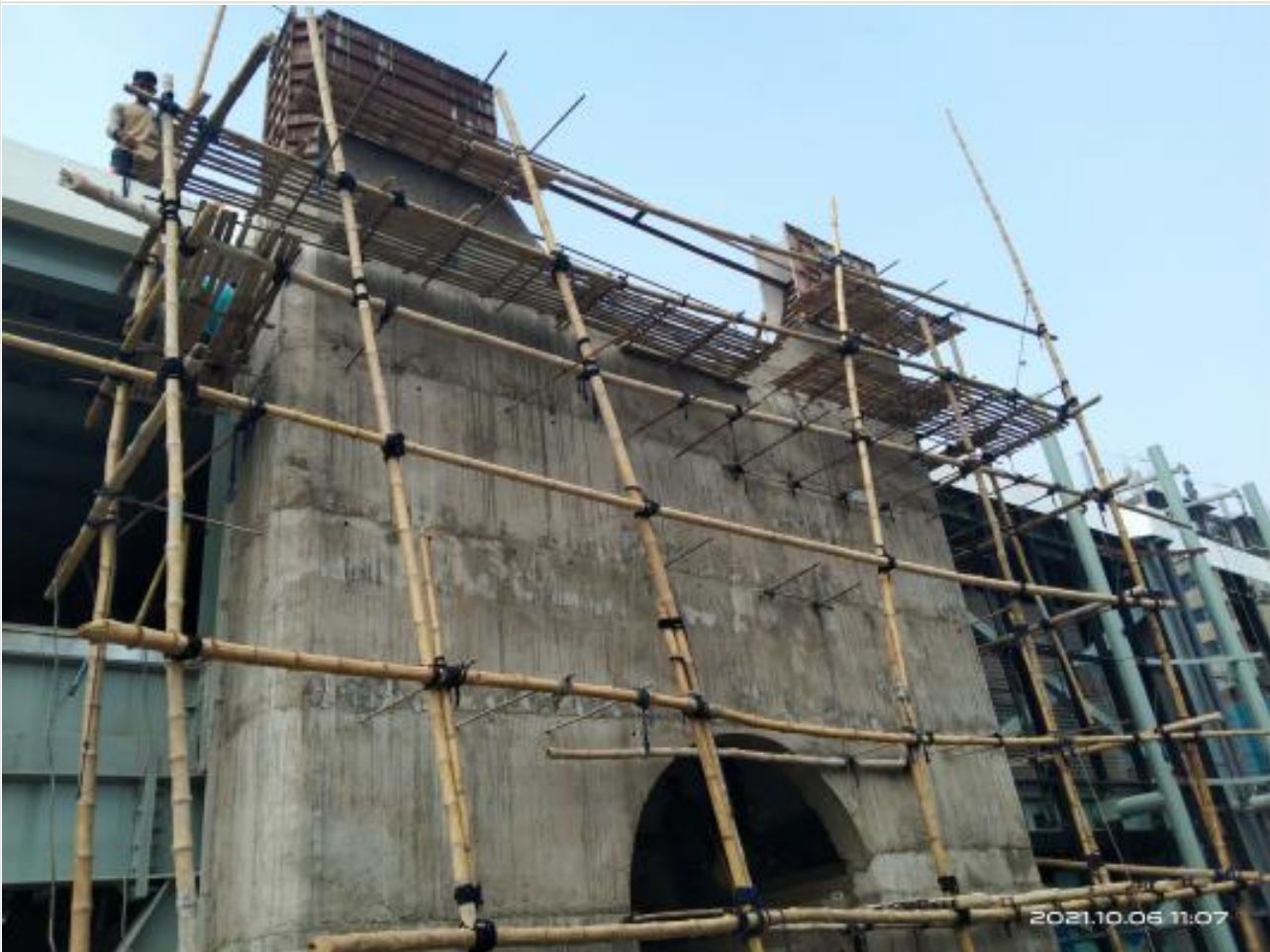
Stair wall casting of stair no. 02 on 06-10-21
