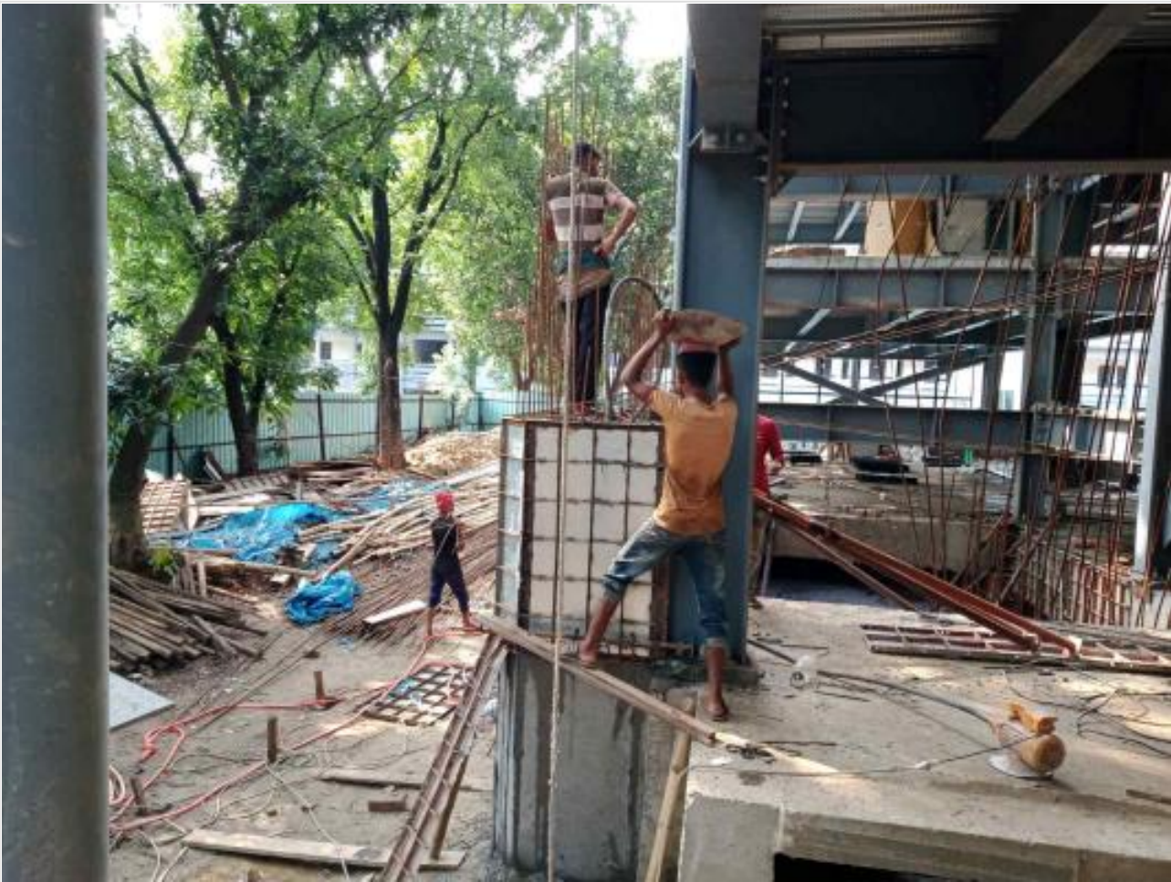
Ground Floor Stair Wall Concreting on 31-05-21
