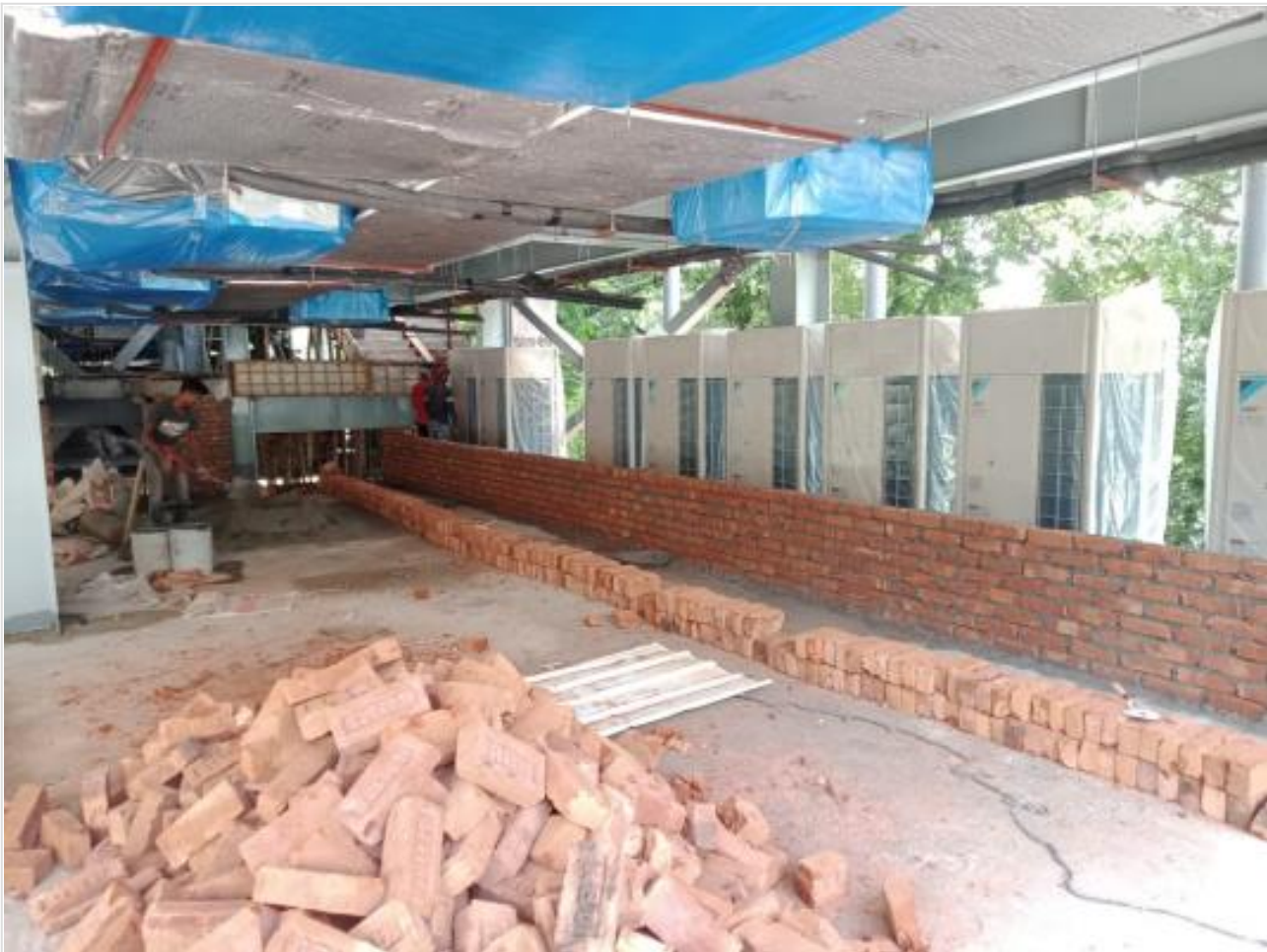
Gr.Floor Mezzanine Brick-Work on 08-07-21
