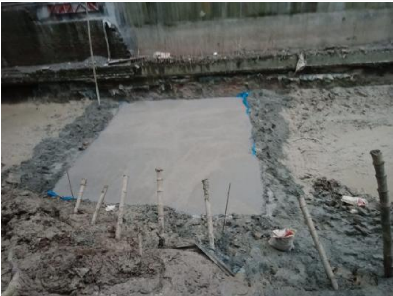
Fire Tank CC Base Casting on 10-09-21
