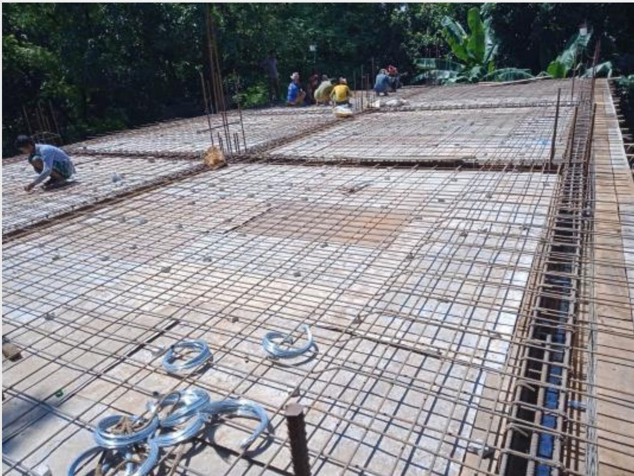
Rod binding work at Generator room slab on 27-09-21
