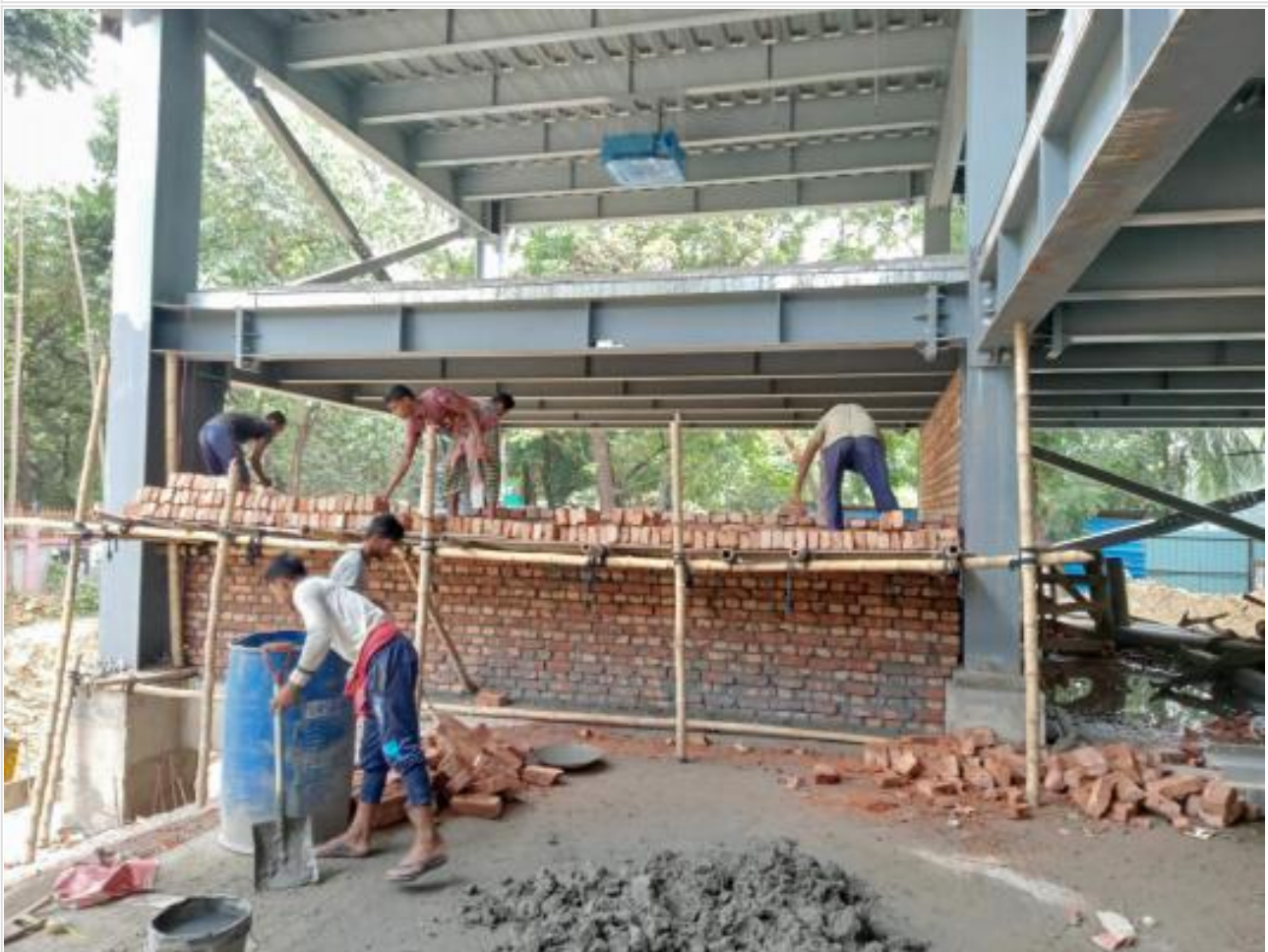
Ground Floor Brick Work on 25-05-21
