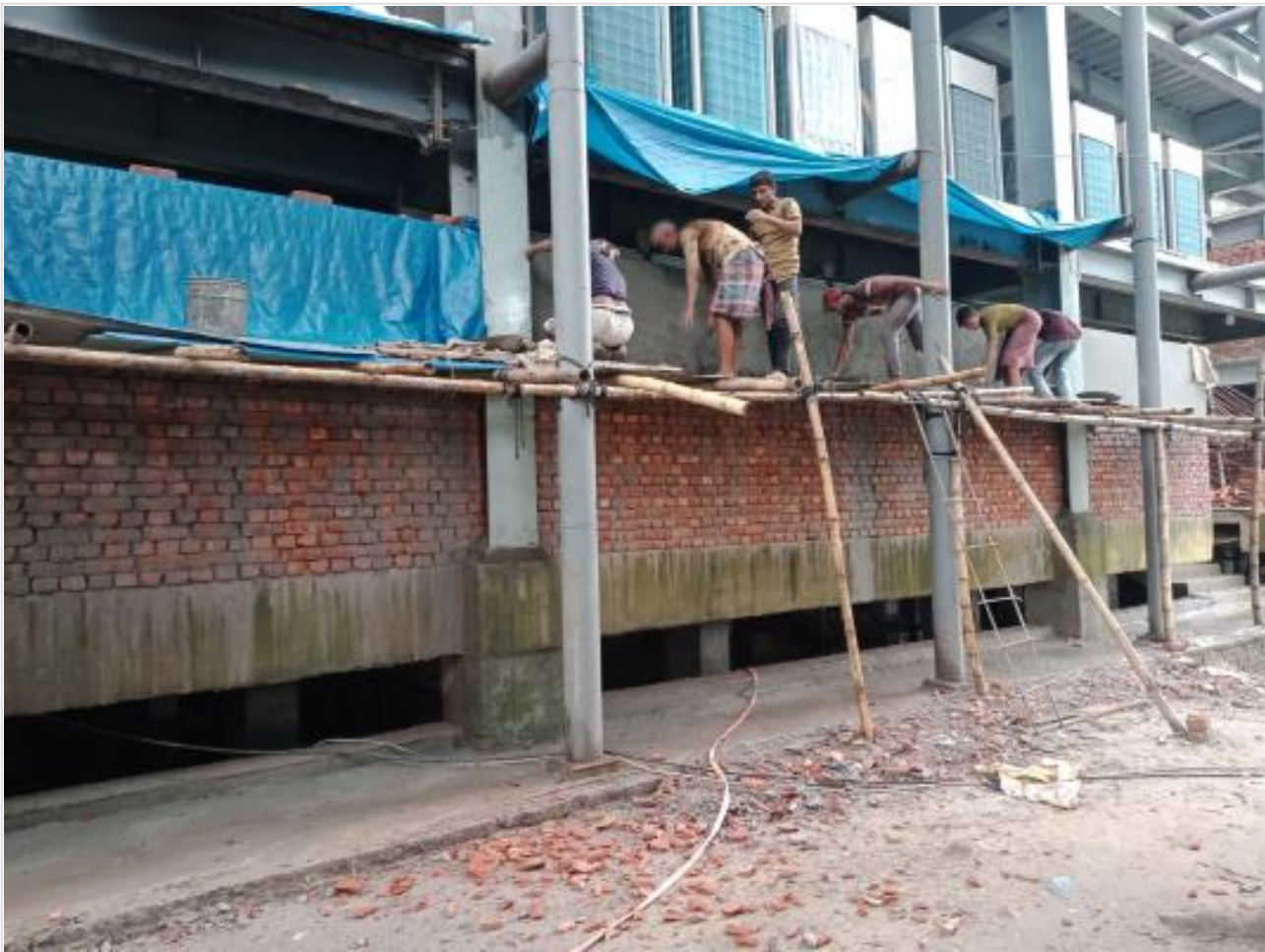
GF Brick wall on 11-08-21
