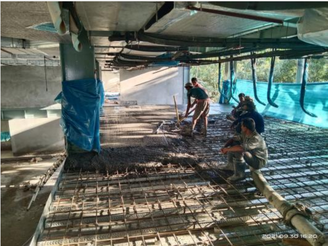
1F Mezzanine Slab Concreting on 30-09-21
