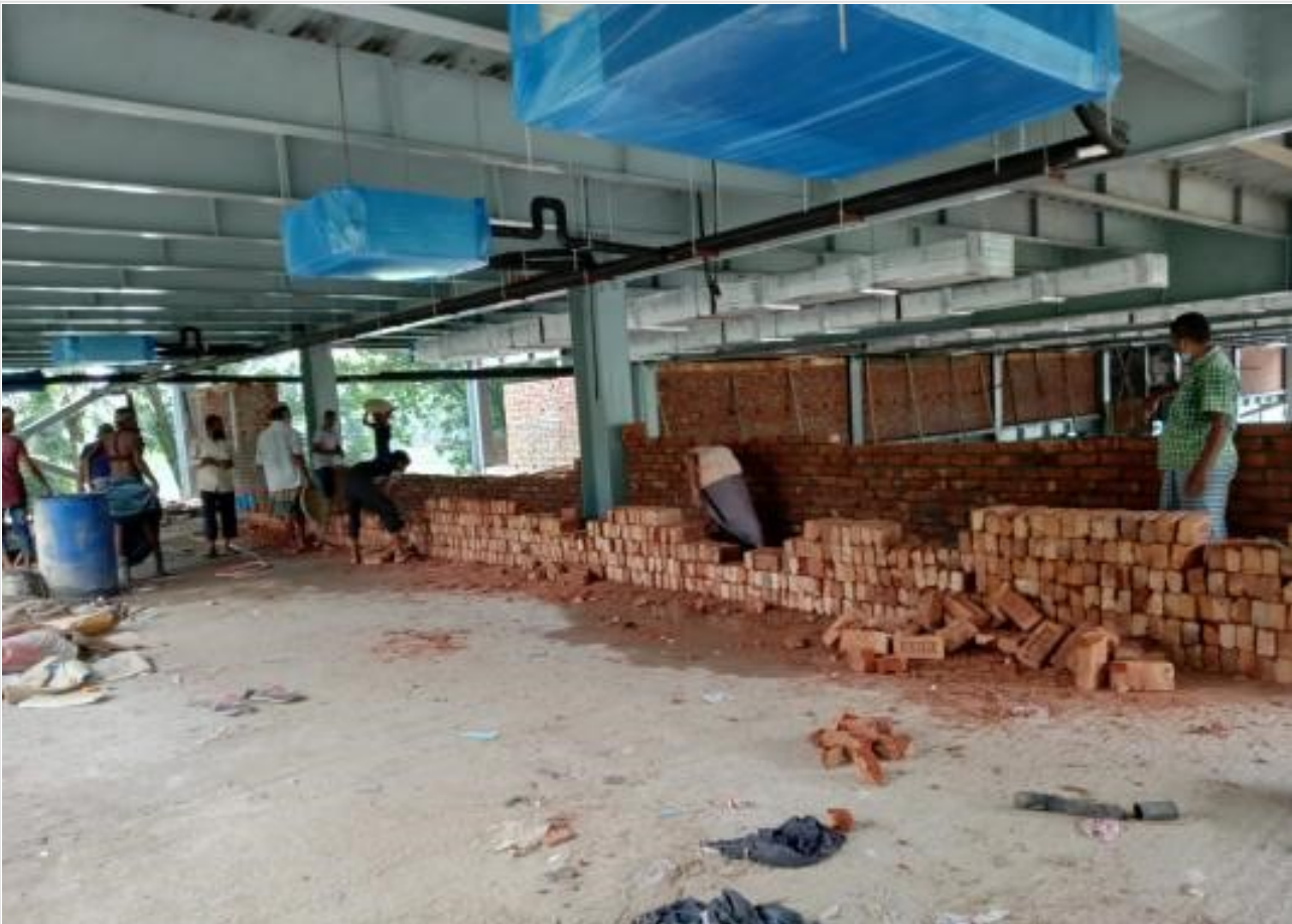
GF mezzanine brick work on 02-08-21
