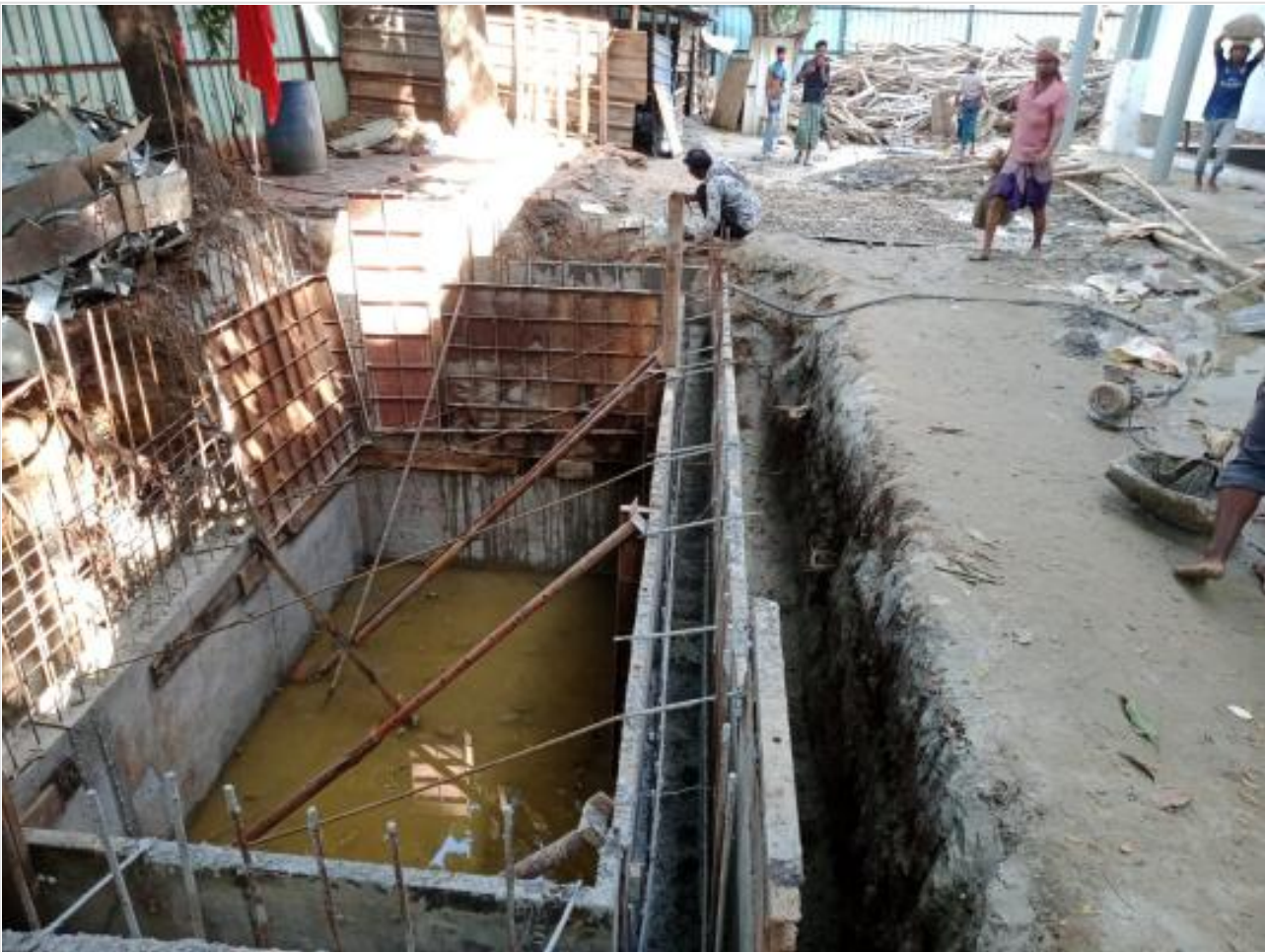
Septic tank wall shuttering on 01-10-21
