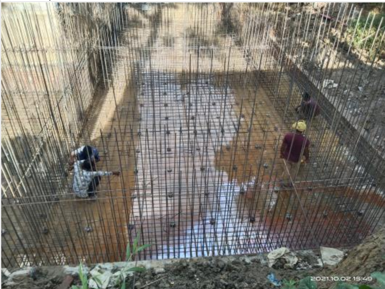
Fire tank base and wall rod binding on 02-10-21
