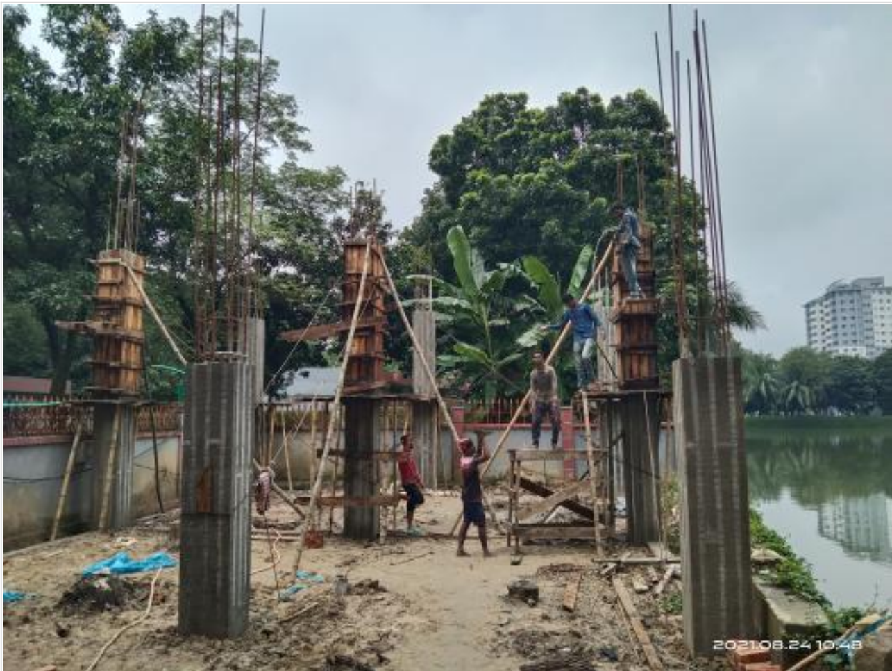
Generator room column casting on 24-08-21
