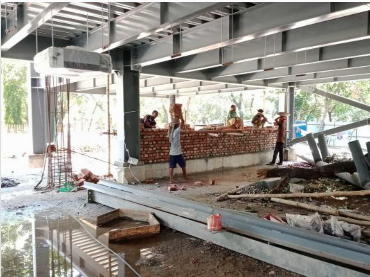
Ground Floor Brick Work on 22-05-21
