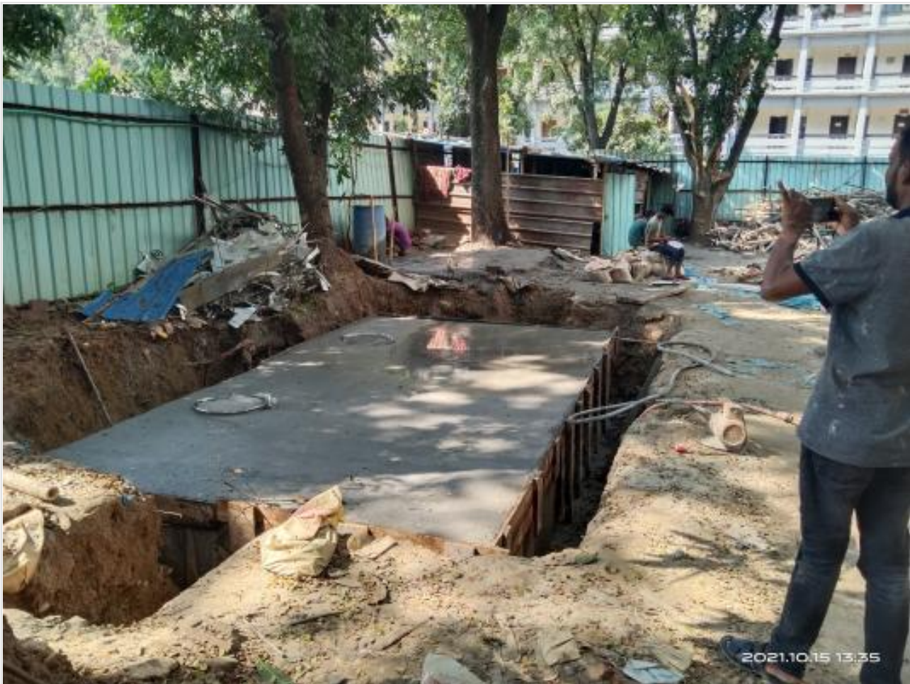
Septic tank top slab casting on 15-10-21
