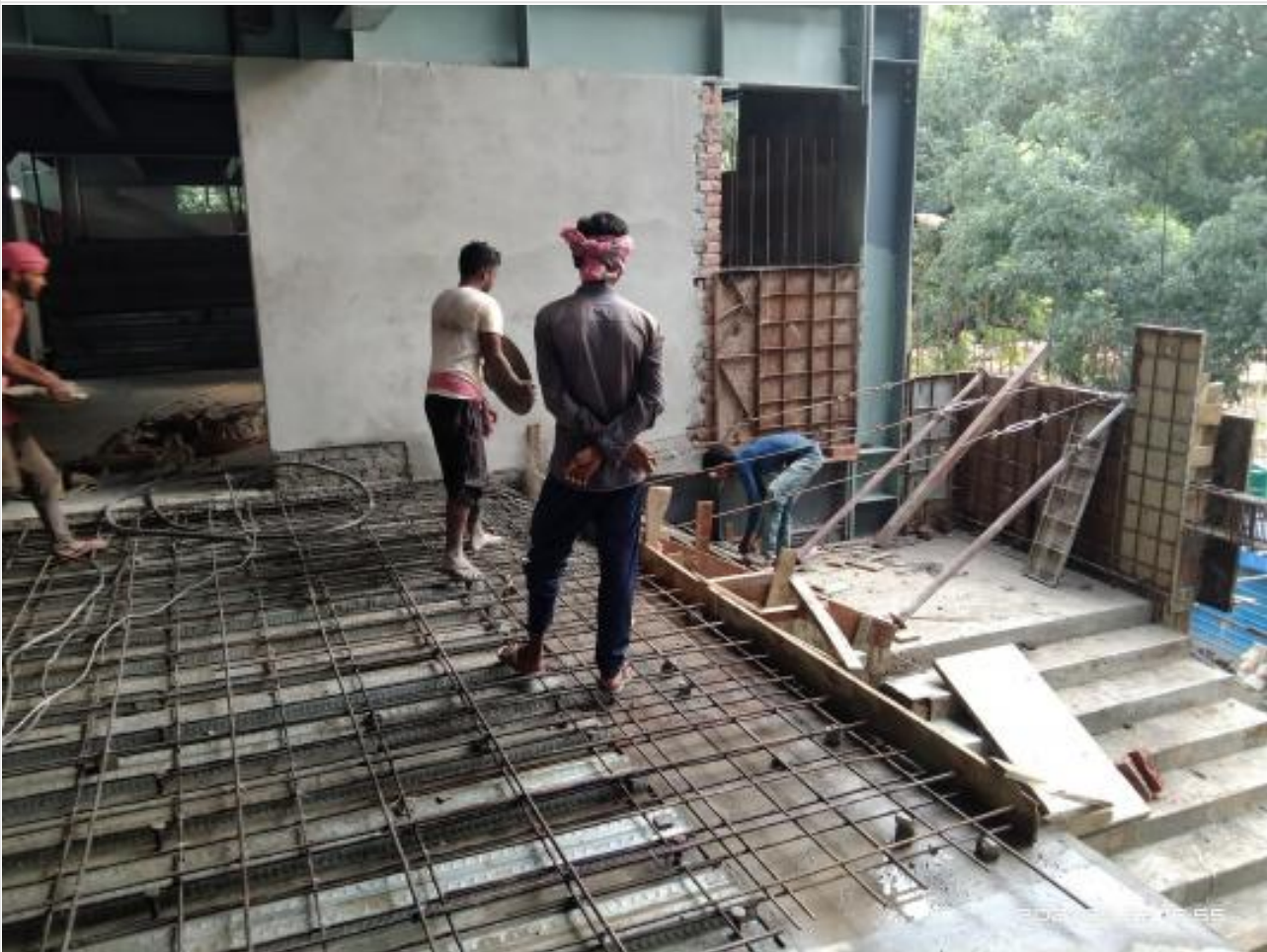
GF Mezzanine stair casting (4-no) on 23-09-21
