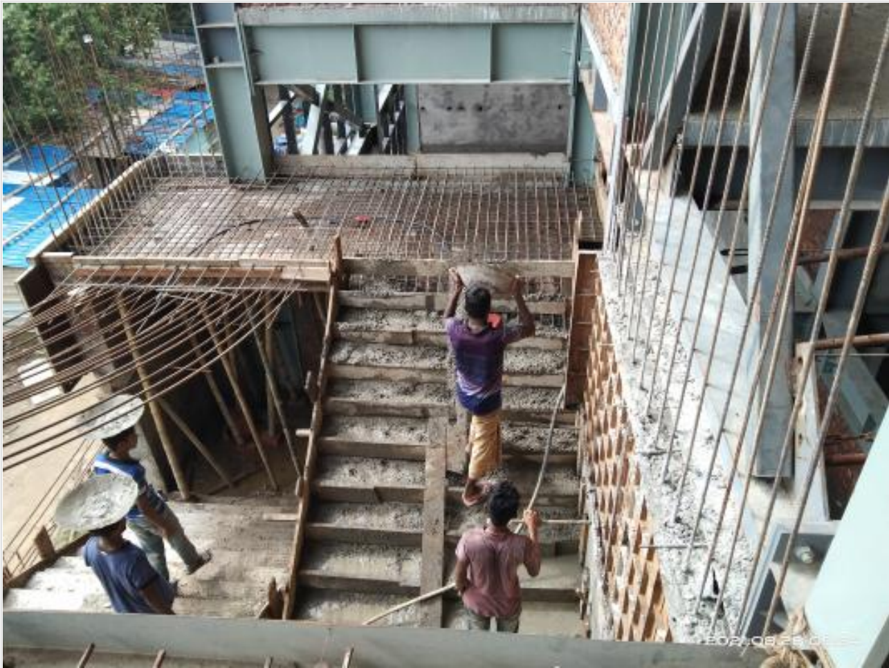
GFM stair casting (stair no. 4) on 28-08-21
