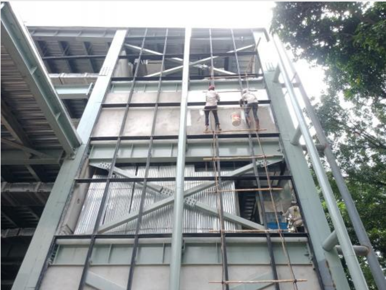
Outside painting work on 19-09-21
