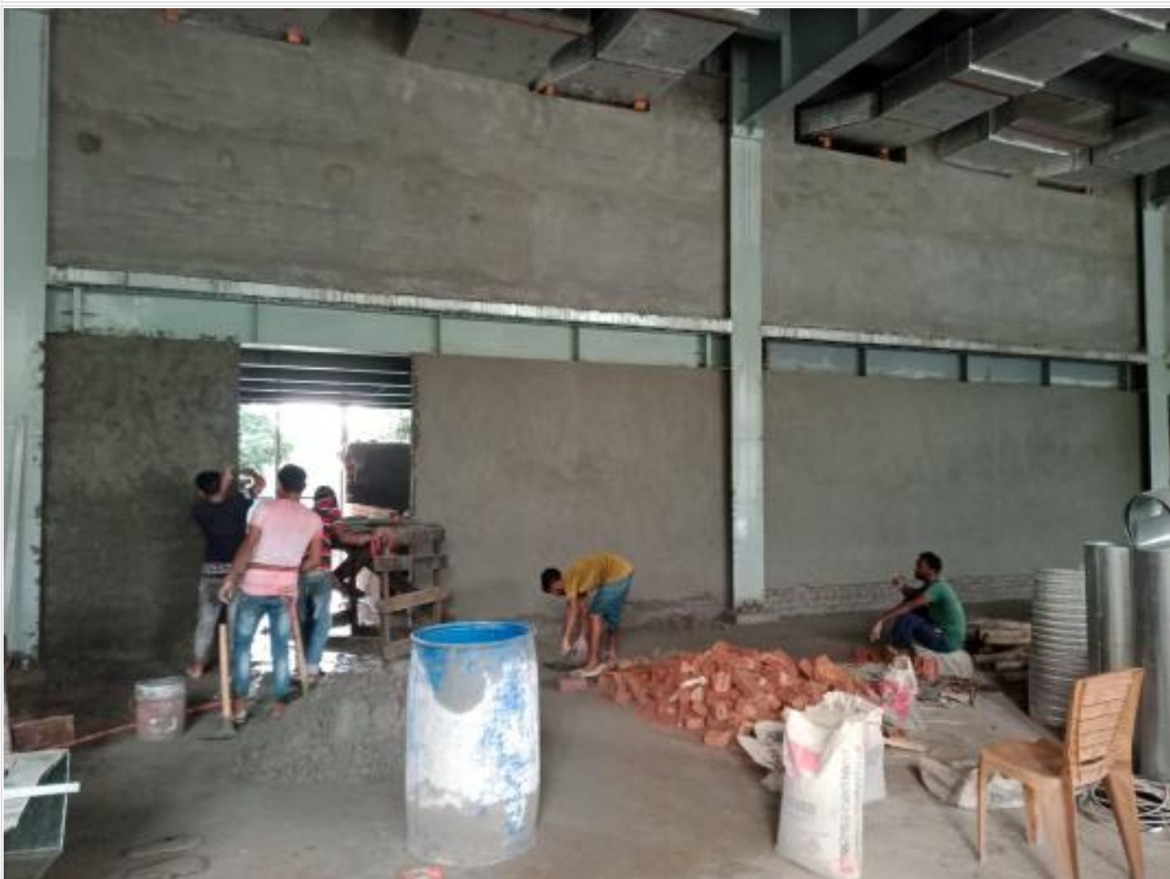
GF plaster work on 13-08-21
