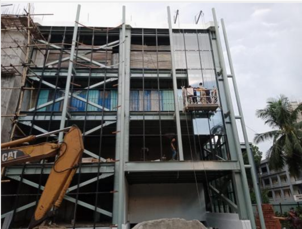
Glass fitting work on 27-09-21
