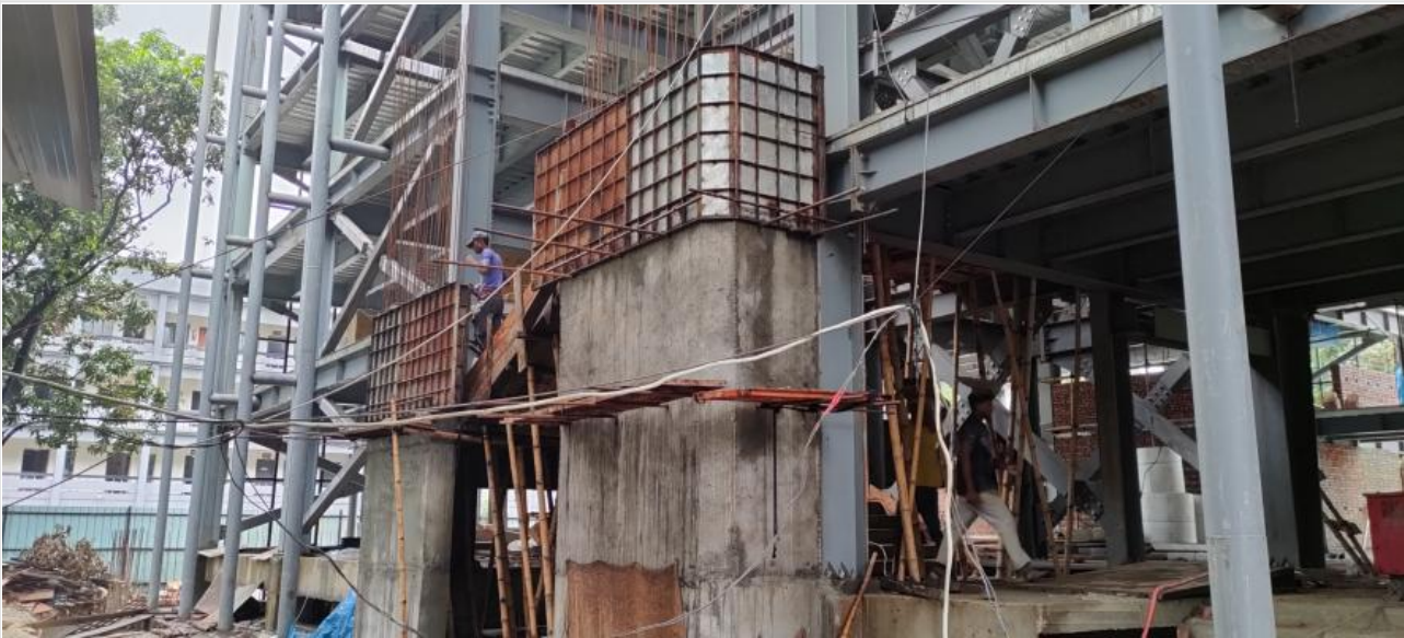
GF Mezzanine Stair Wall Concreting on 16-06-21
