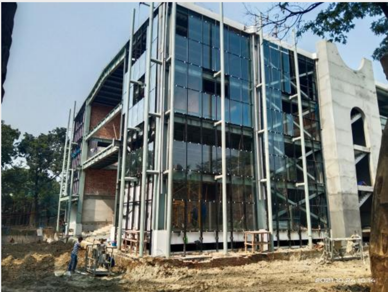
South East corner glass fitting on 24-10-21
