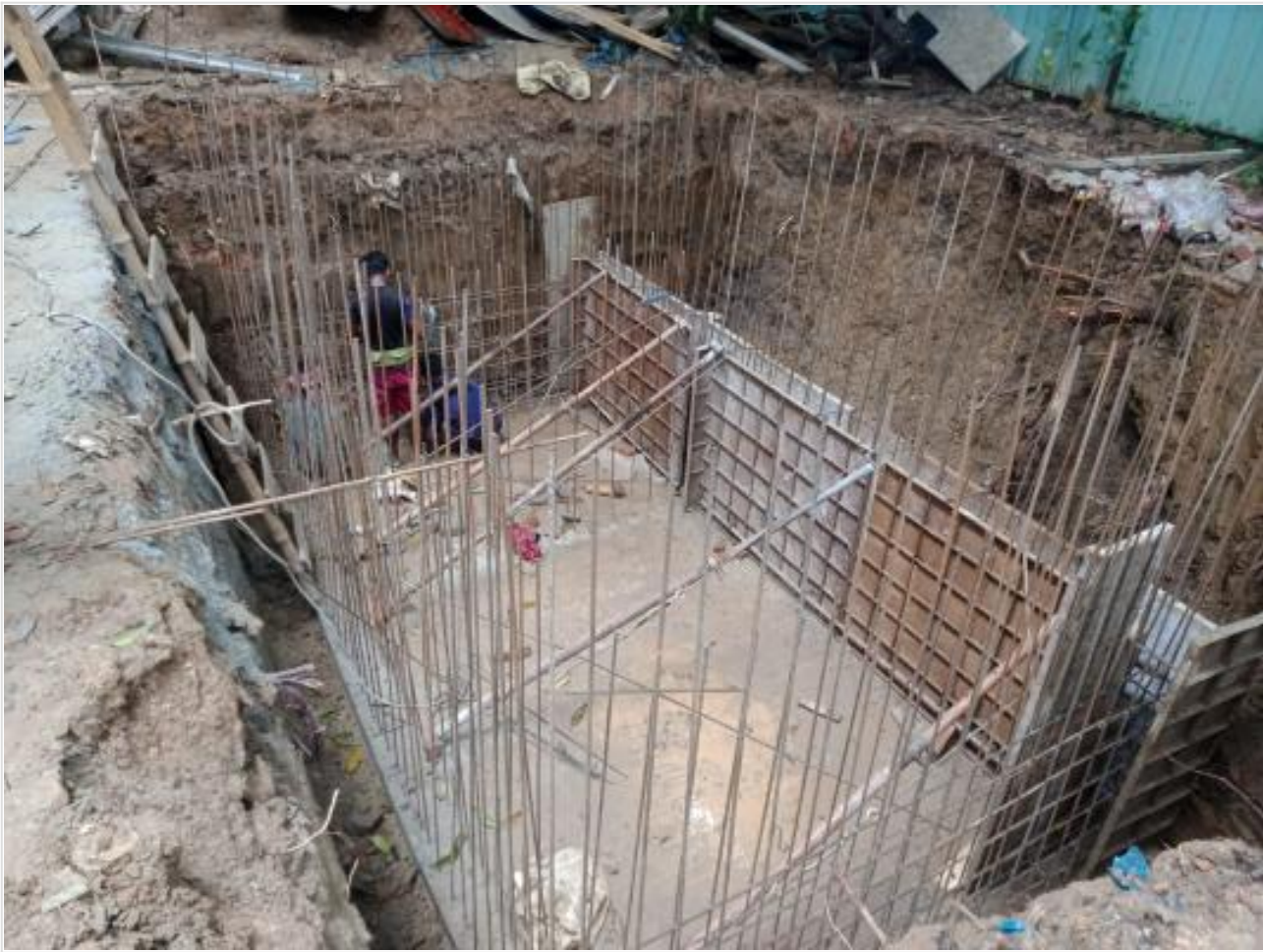
Spitic tank RCC Base casting on 17-09-21
