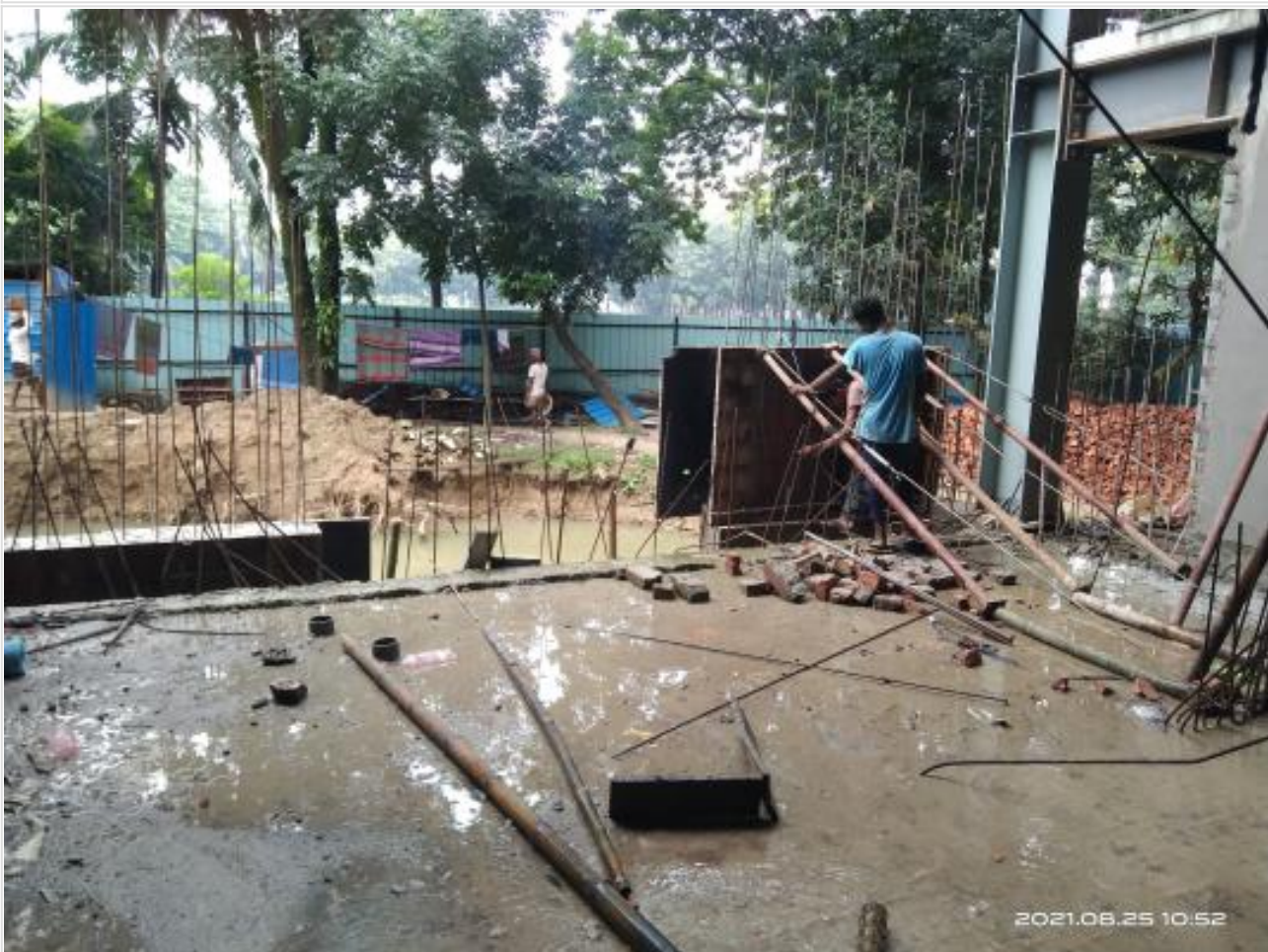
GG stair wall (stair no-4) on 25-08-21
