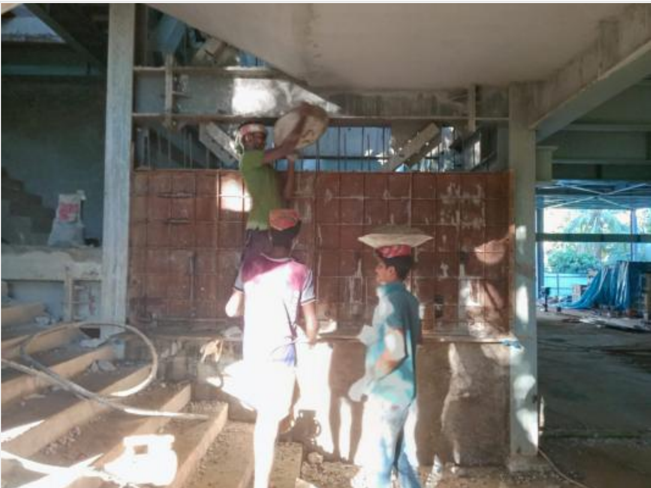
GF Lift wall Casting on 31-08-21
