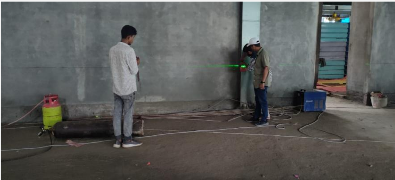
False ceiling level marking on 11-09-21
