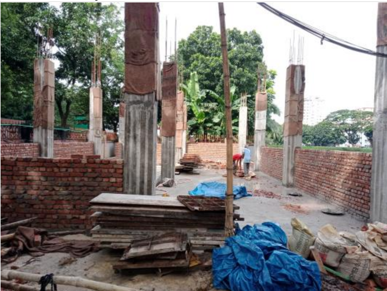
Generator room brick work on 10-09-21
