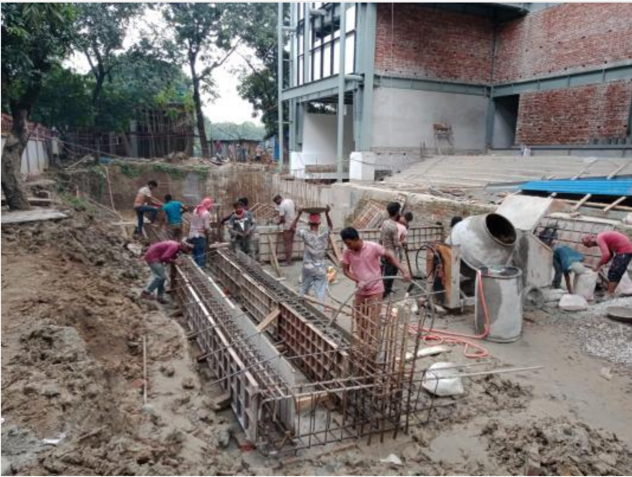
South canopy GB casting on 14-10-21
