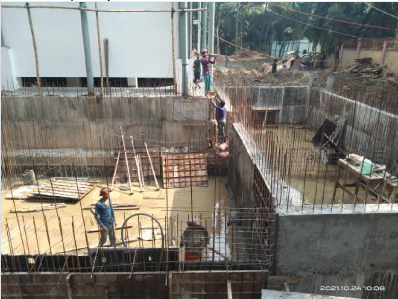
Fire tank wall casting on 24-10-21
