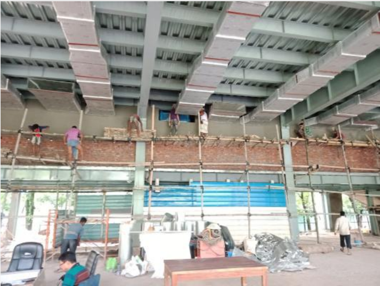
GF Mazzanine wall plaster on 04-08-21
