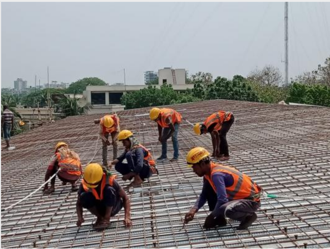
Roof Slab Re-bar Work on 01-05-21
