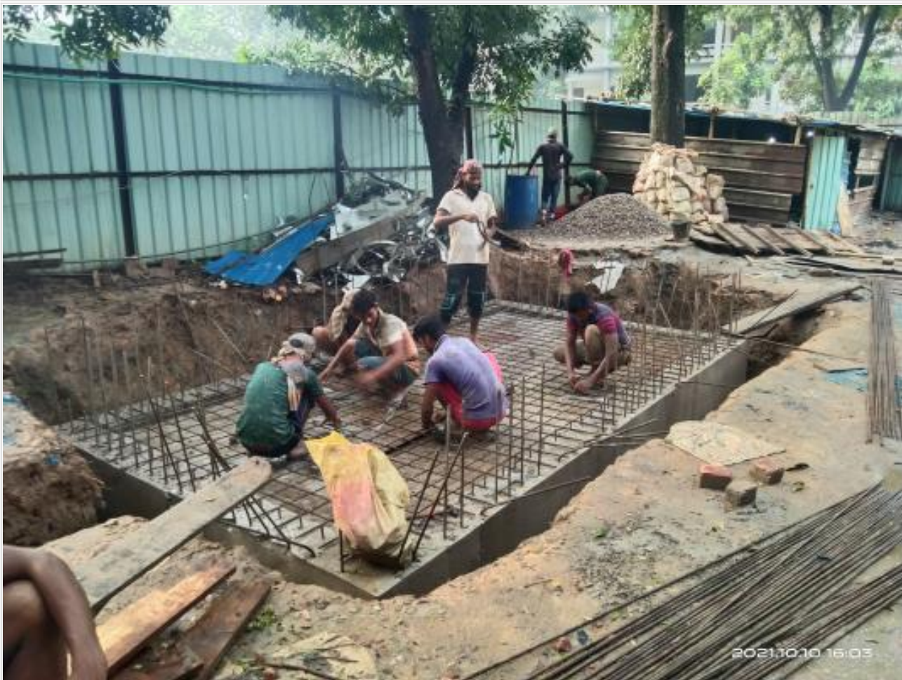
Septic tank top slab rod binding on 10-10-21
