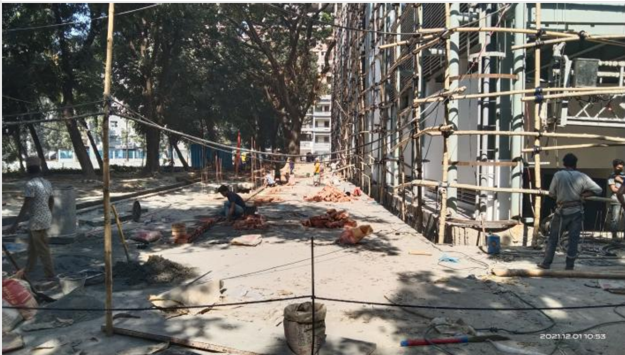
Road Construction on 30-11-21
