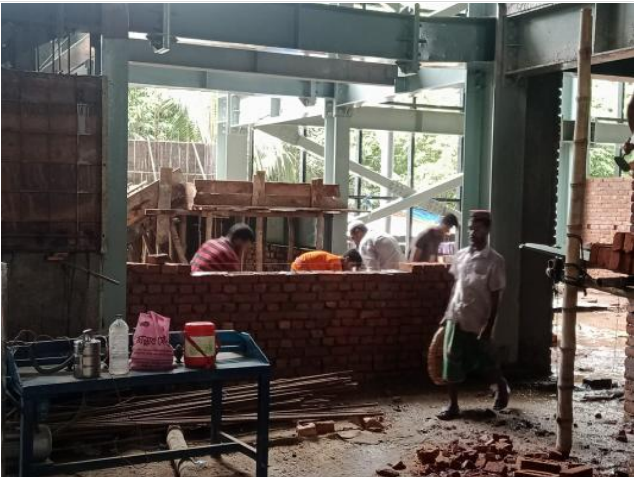
GF brick work on 15-08-21
