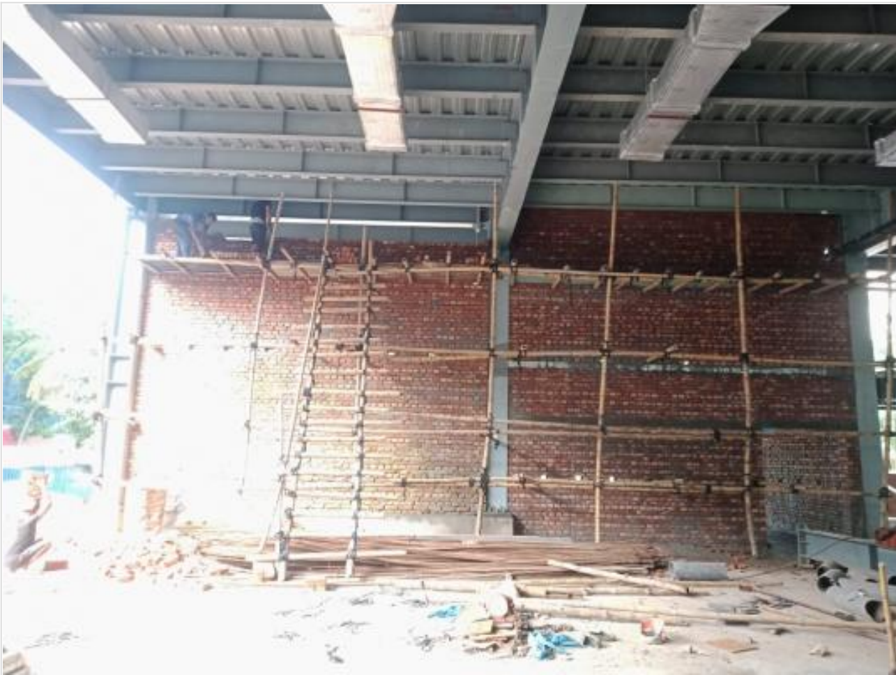
Gr.Floor Mezzanine Brick Work on 23-06-21
