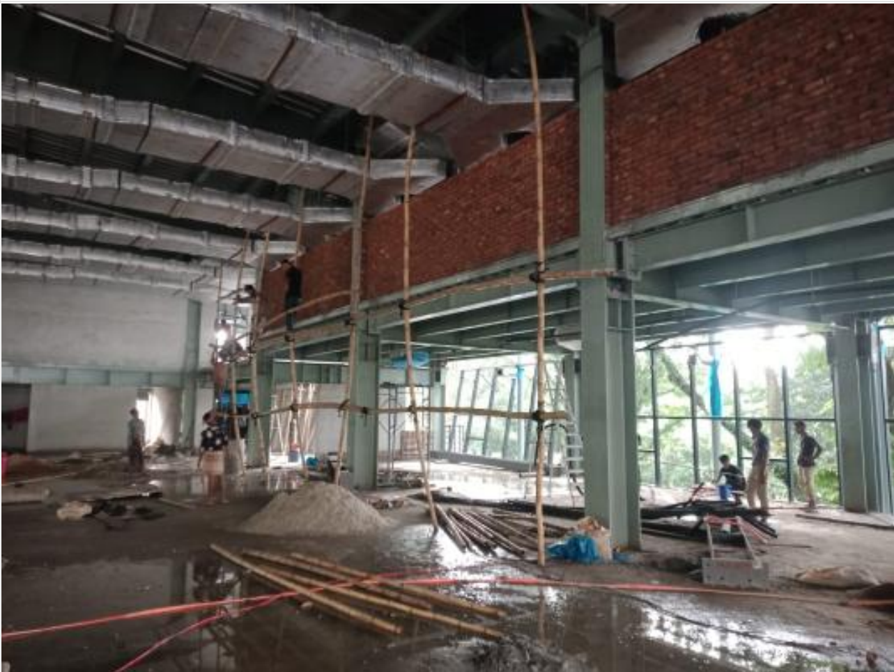
FFM brick wall plaster on 08-10-21
