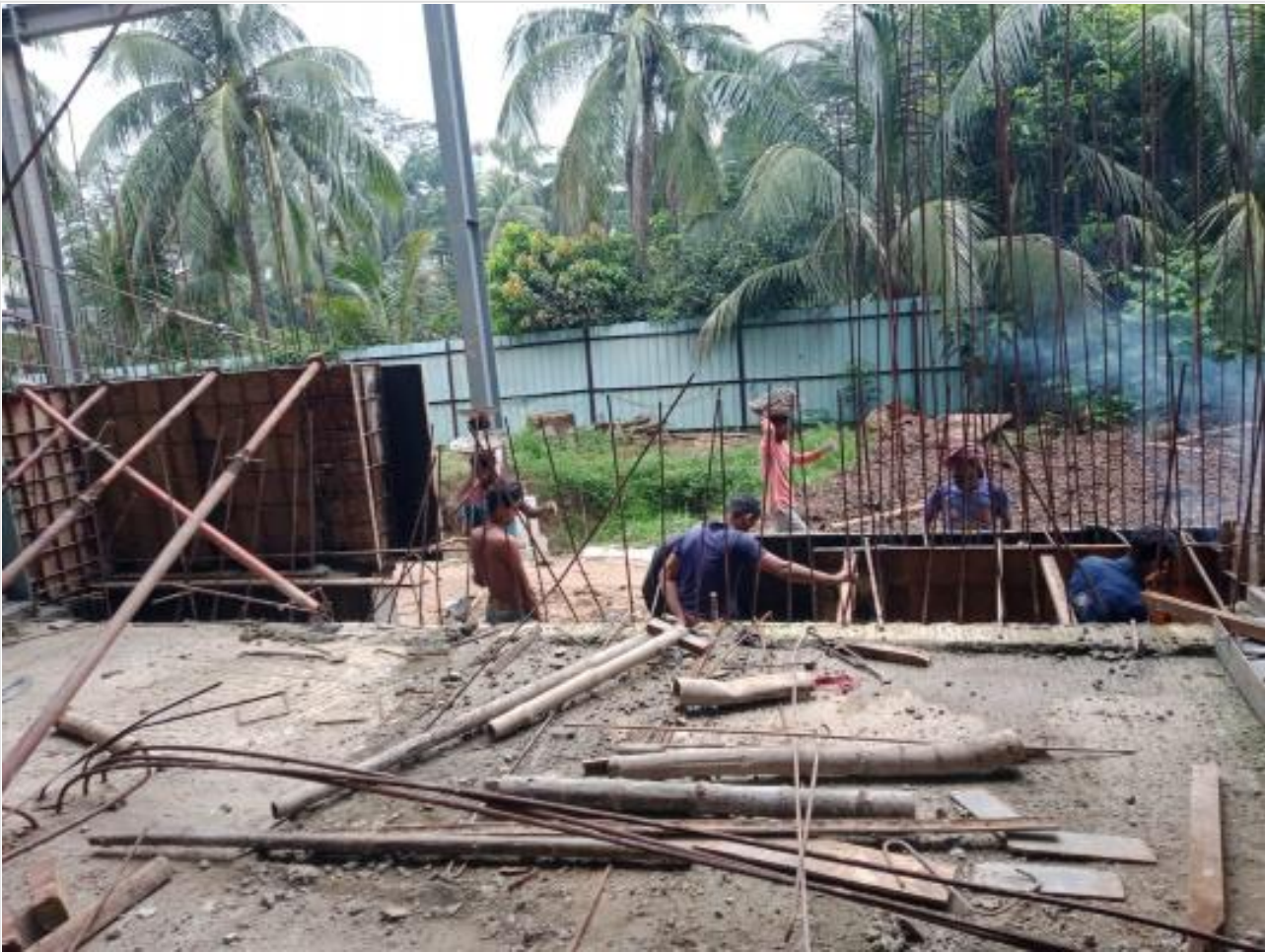
GF stair work (stair no-3) on 10-08-21
