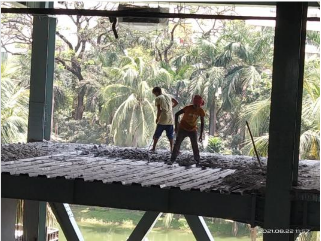
GF Mezzanine floor dismantling on 22-08-21
