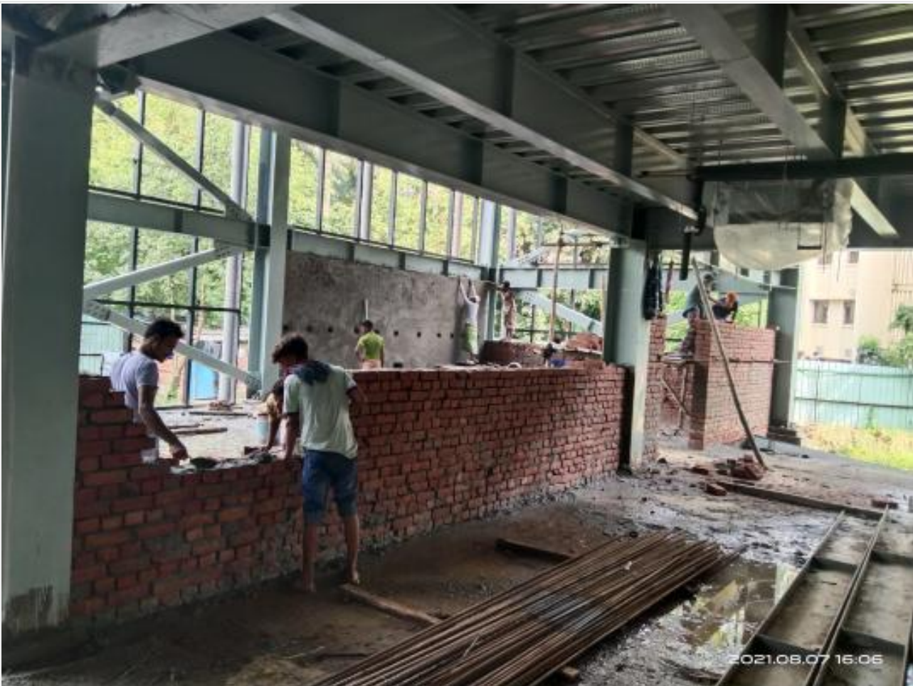
GF brick and plaster work on 07-08-21
