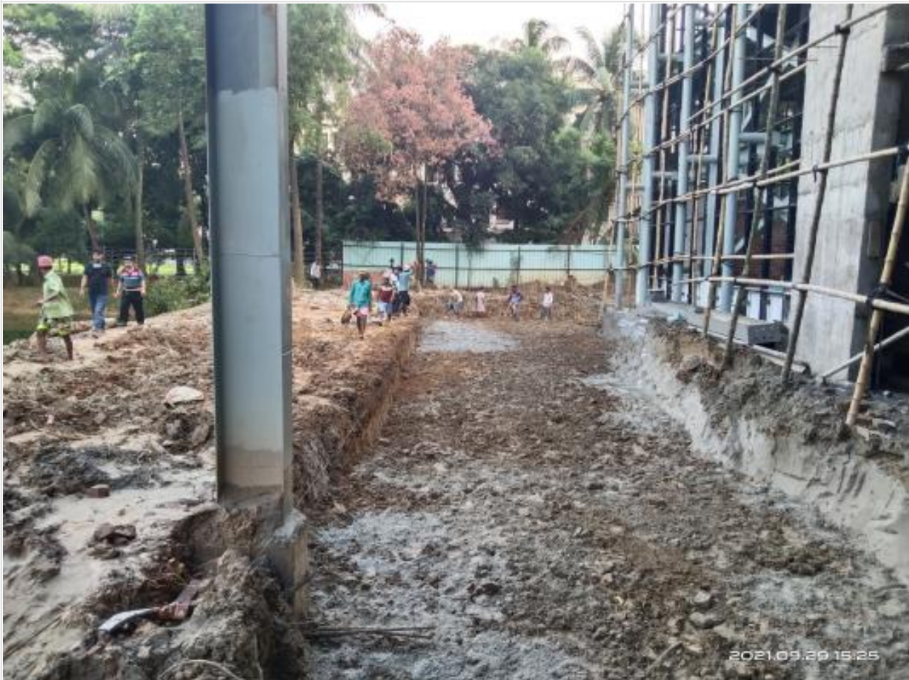
Preparation of subgrade bed of road on 29-09-21
