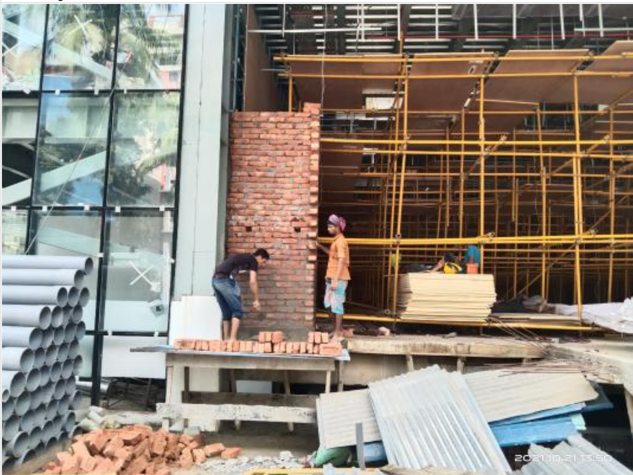
North side front brick work on 21-10-21
