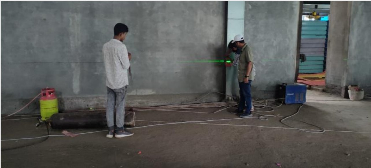
False ceiling level marking on 11-09-21
