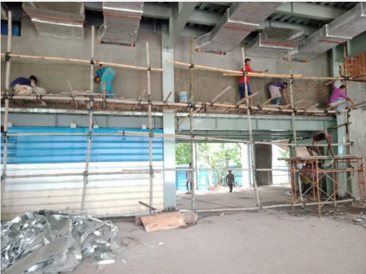
Ground Floor Mezzanine Plastering on 06-08-21
