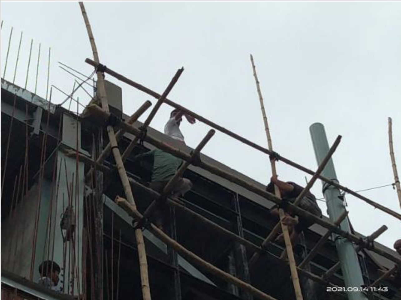
Gutter plaster work on 14-09-21
