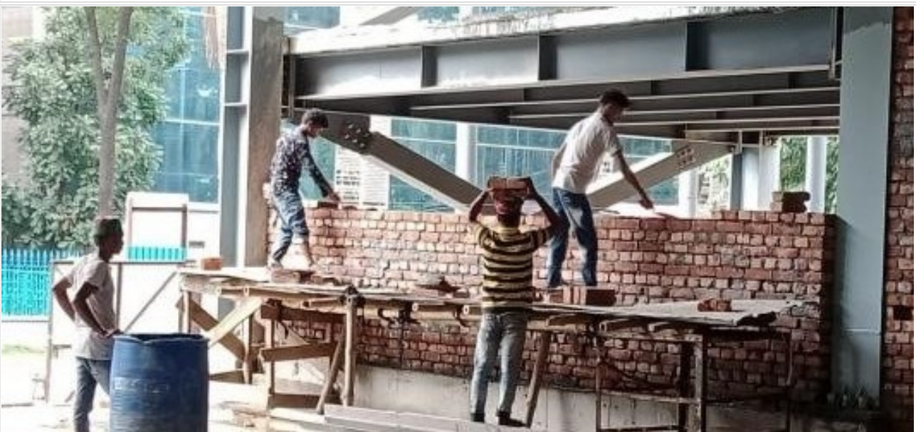
Ground Floor Brick Work on 19-05-21
