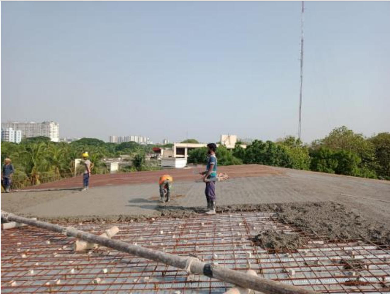
Roof Slab Concreting on 06-05-21
