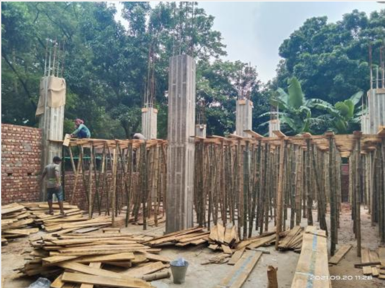
Sub-Station and Generator room staging f on 20-09-21
