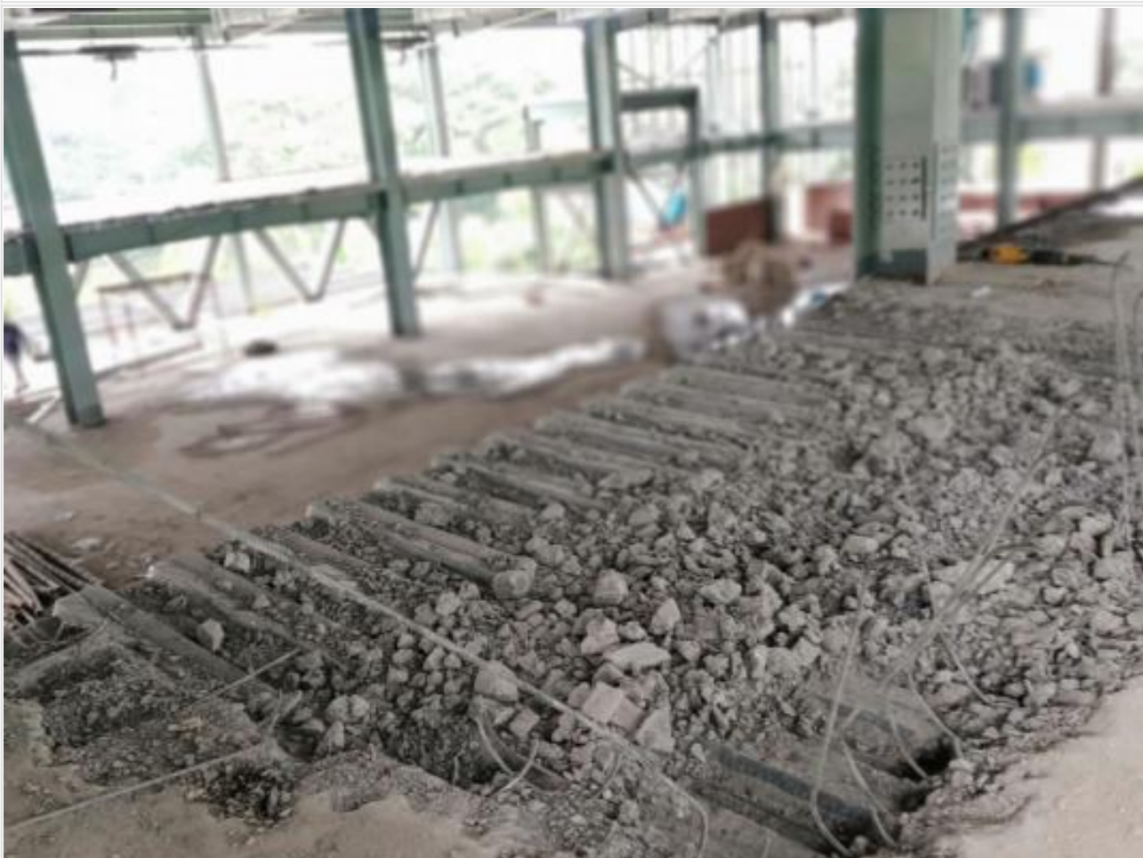
FF Mezzanine floor dismantling work on 18-08-21
