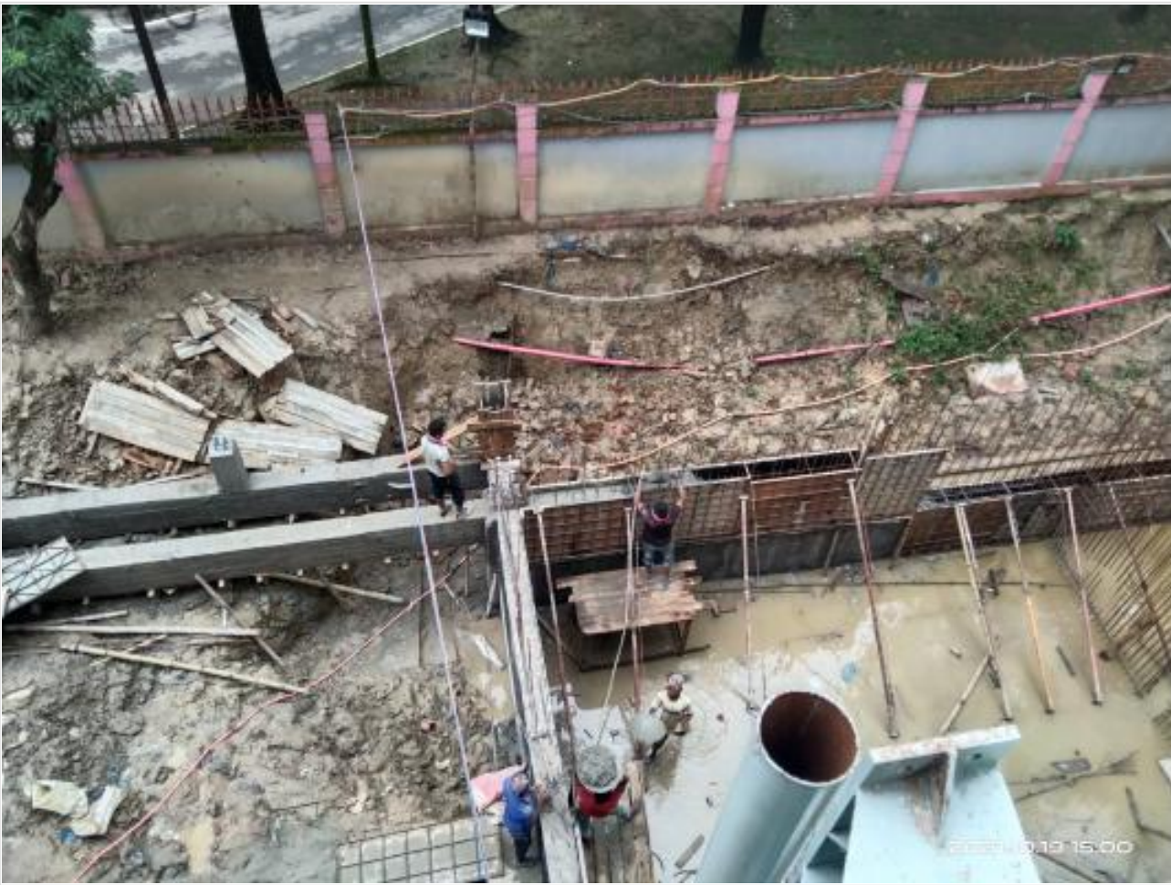
Fire Tank wall casting on 19-10-21
