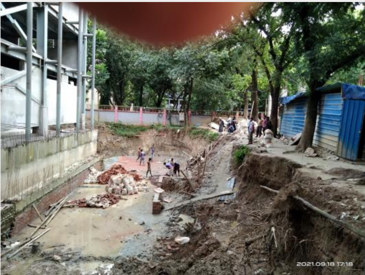
Fire tank cc work on 18-09-21
