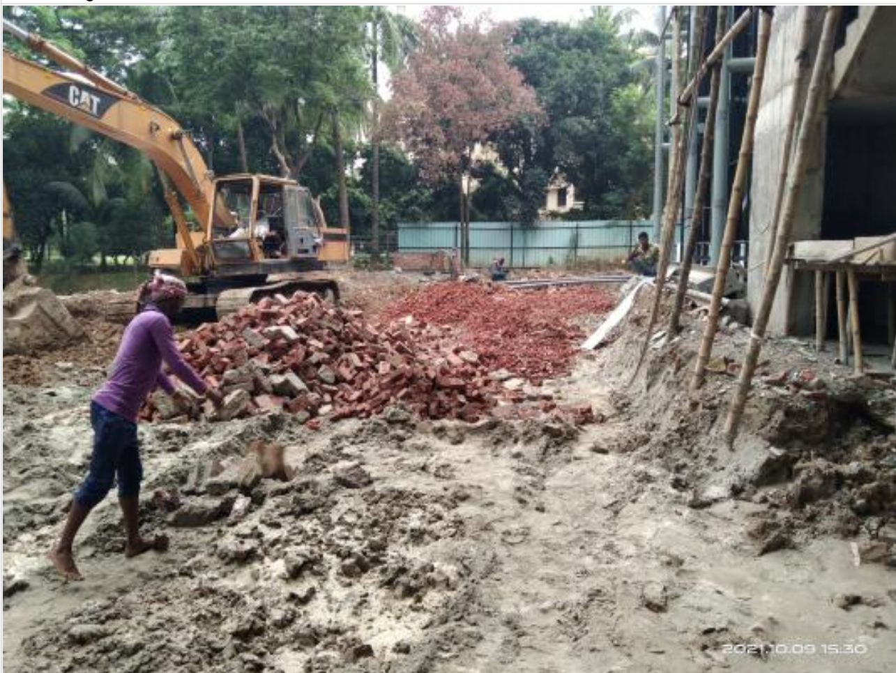
Road work on 09-10-21
