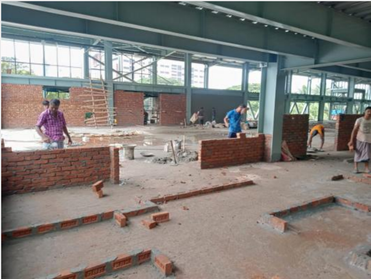
FF brick work on 18-08-21
