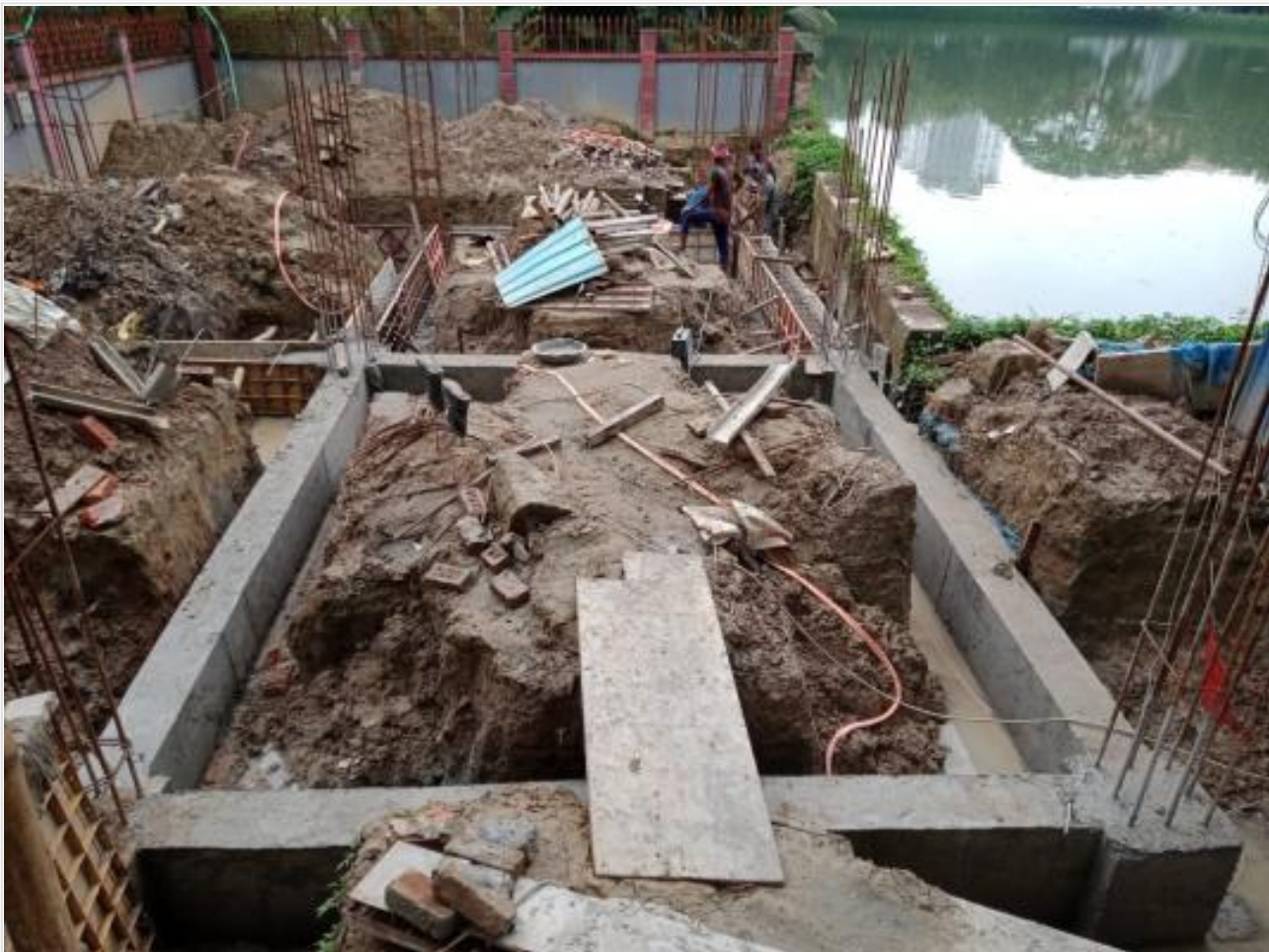
Substation Grade Beam Concreing on 09-08-21
