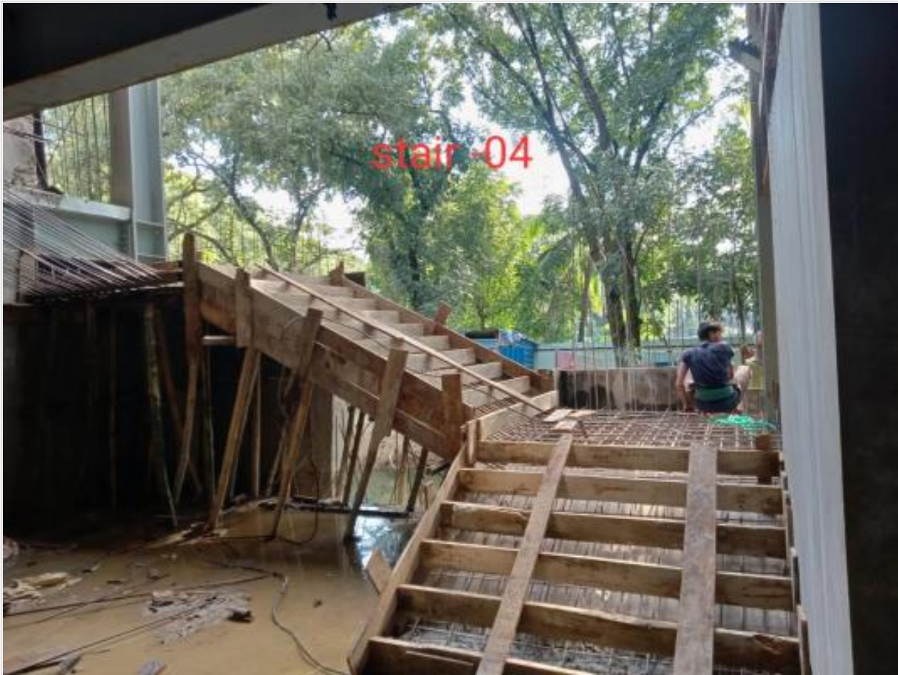
GF Stair casting on 31-08-21
