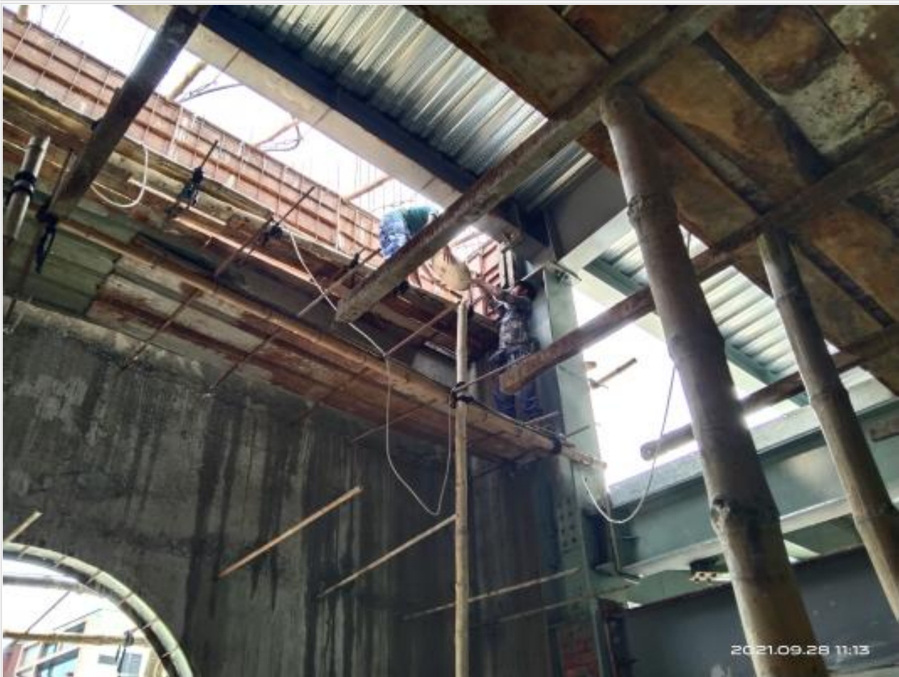
Stair wall casting on 28-09-21
