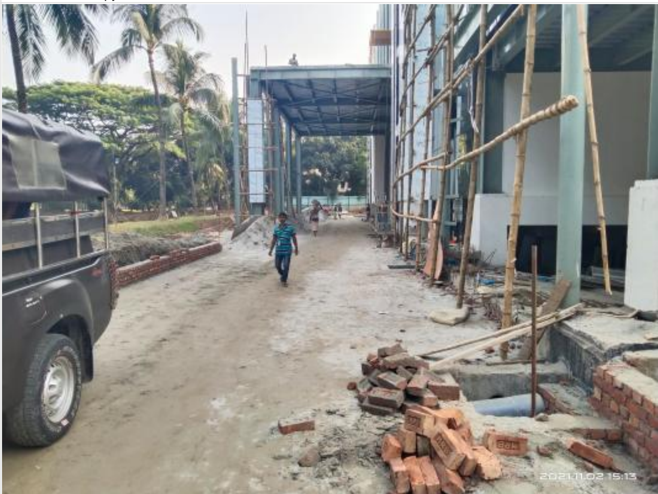
Road sub-base work on 31-10-21
