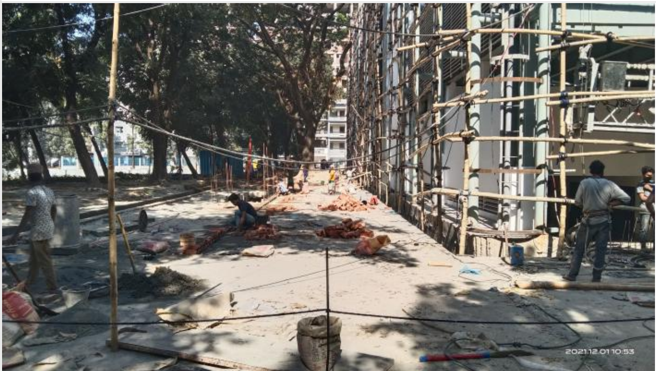
Road Construction on 30-11-21
