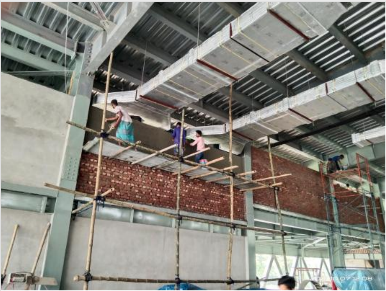
FFM wall plaster on 07-10-21
