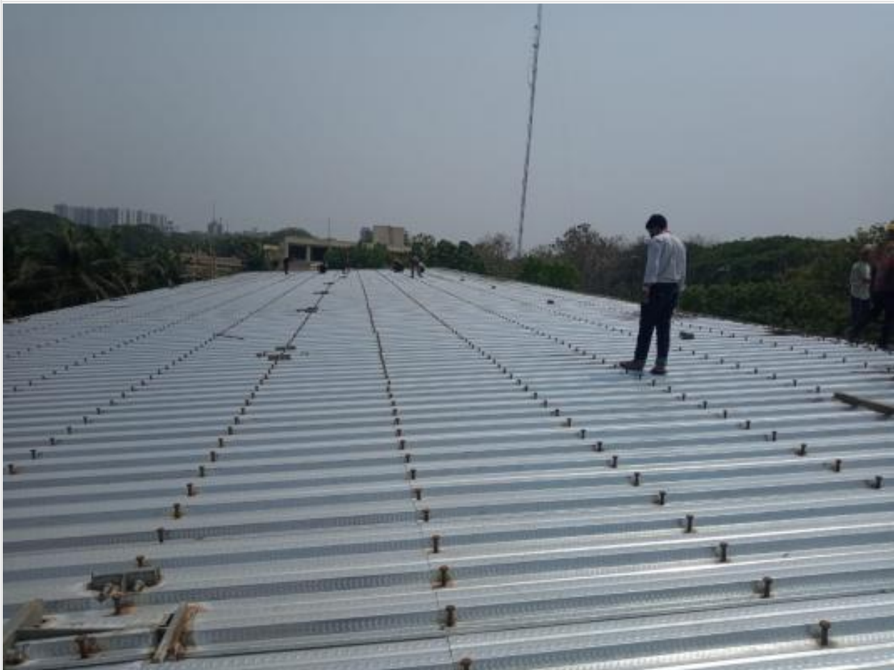
Roof Top Decking on 05-04-21
