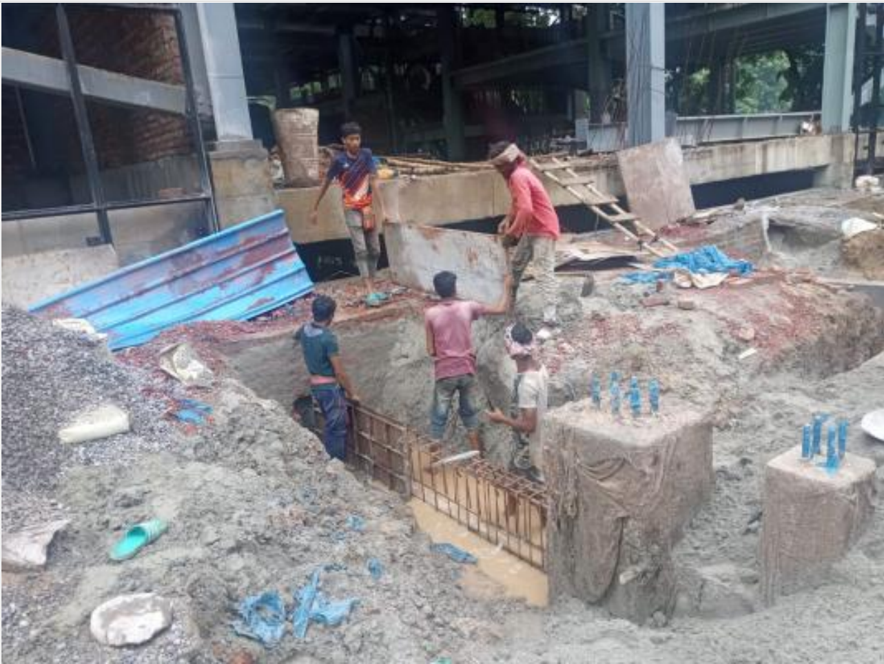
Porch Grade Beam Beam Shuttering on 01-07-21
