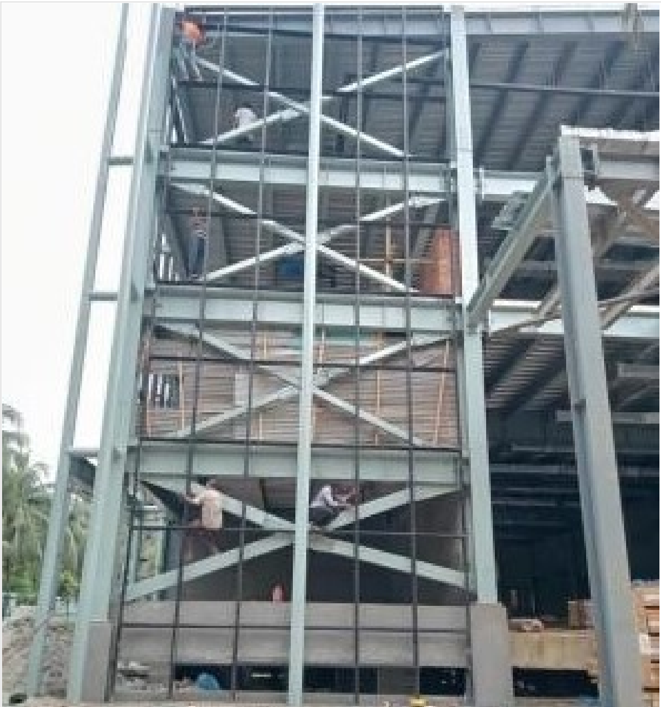
Out side glass frame cleaning on 13-08-21
