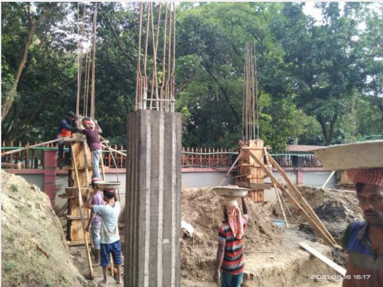
Generator and substation column casting on 16-08-21
