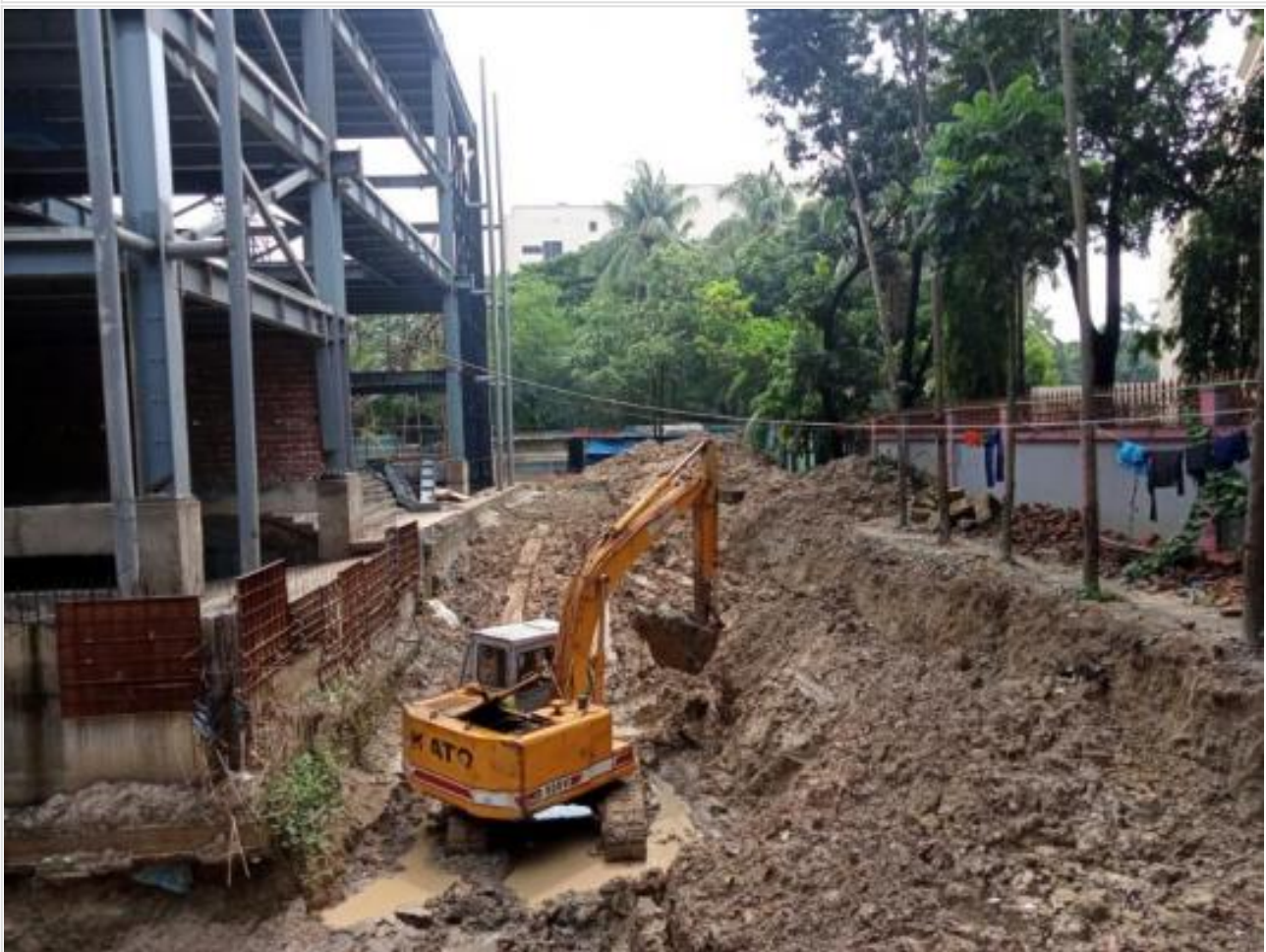
Fire water reservoir excavation on 07-06-21
