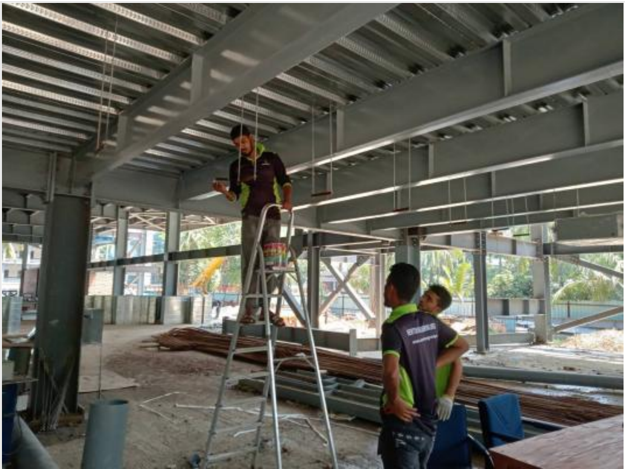
AC Duct Hanging on 22-05-21
