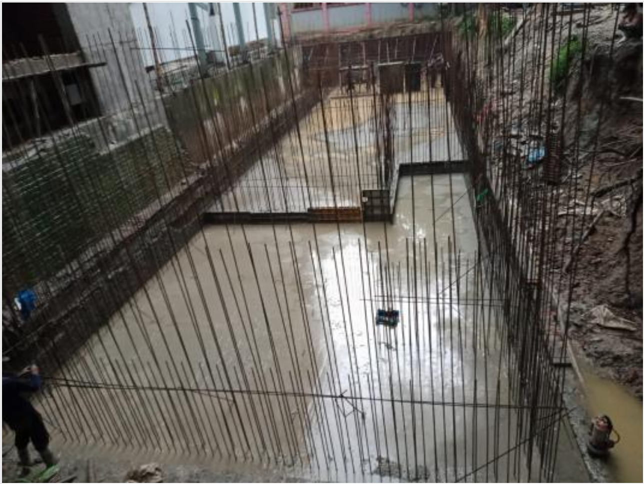
Fire Tank base casting on 20-10-21
