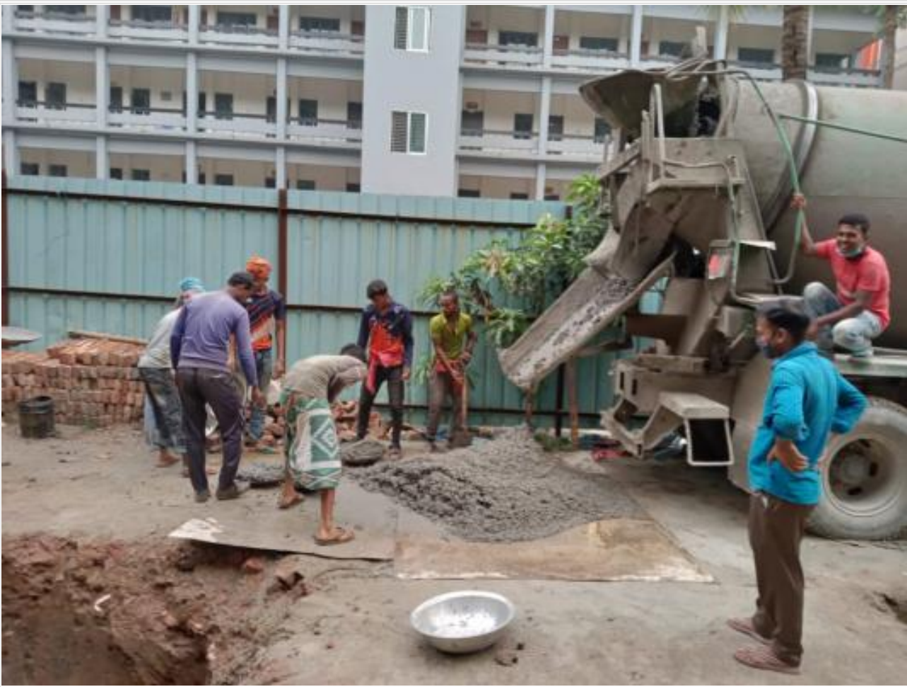
Canopy Base Concreting on 03-05-21
