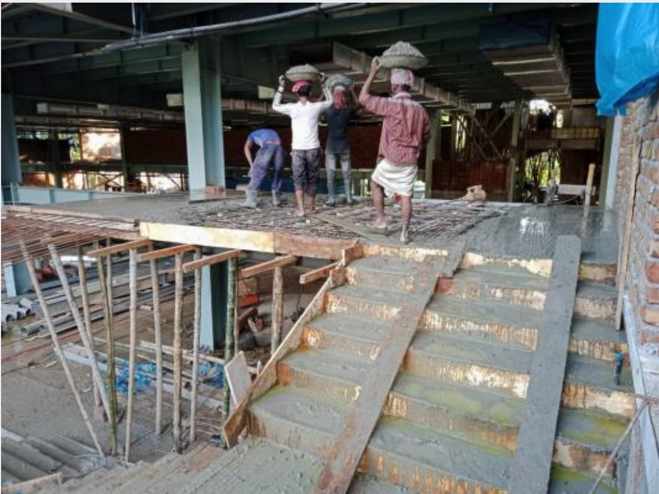
Gr.Floor 3-Flight Stair Concreting on 08-07-21
