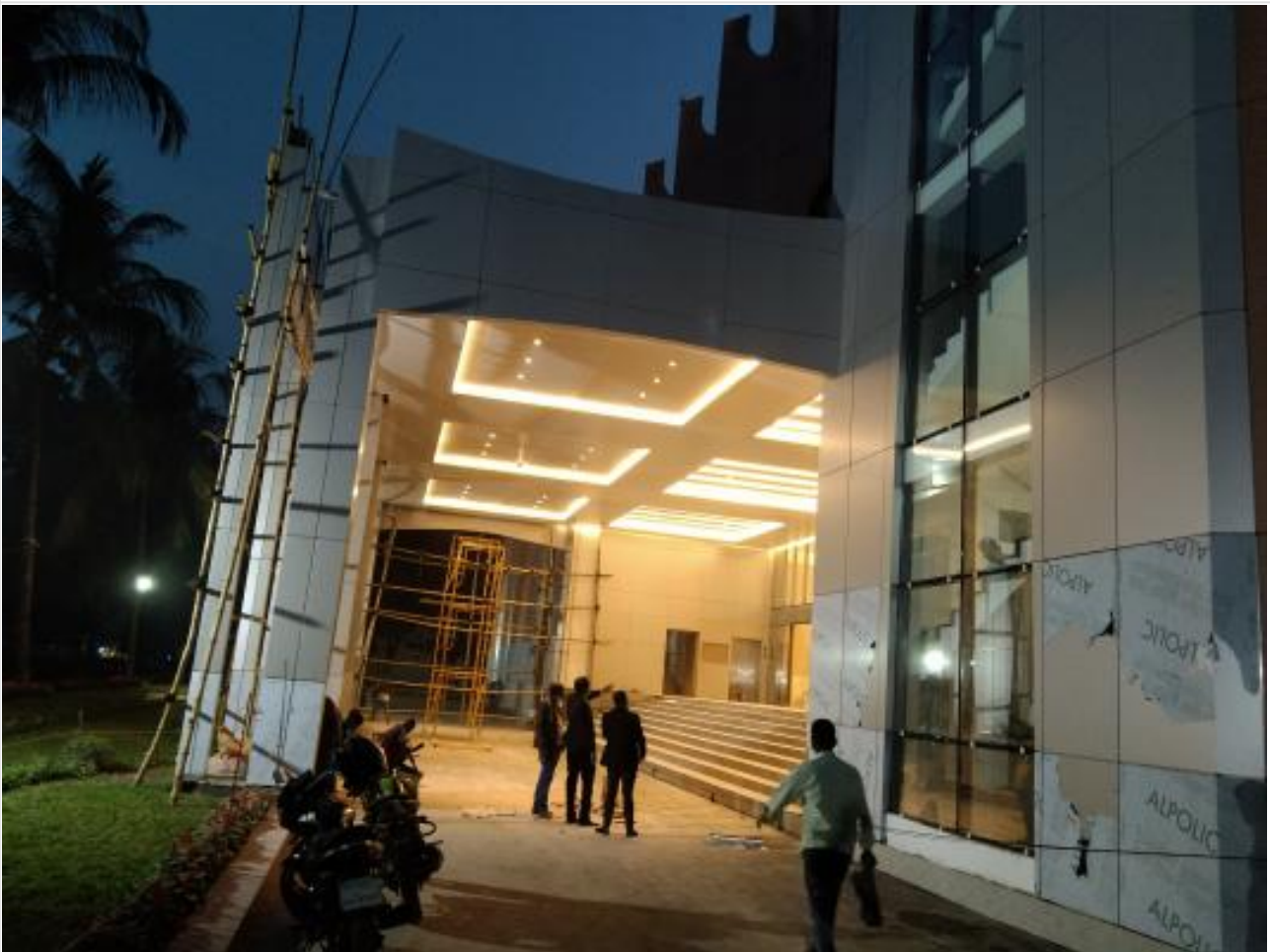
Interior work on 15-12-21
