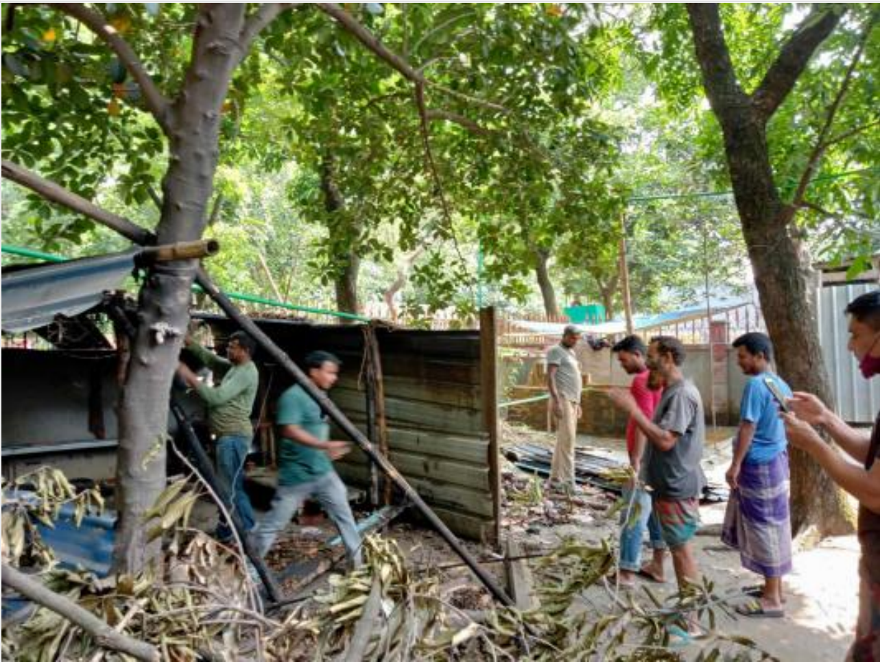
Clearing for Substation Room Layout on 02-06-21
