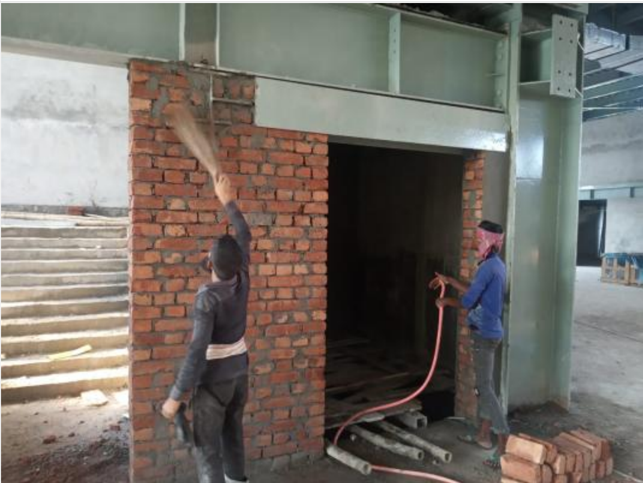
1st Floor lift door side brick wall on 24-09-21
