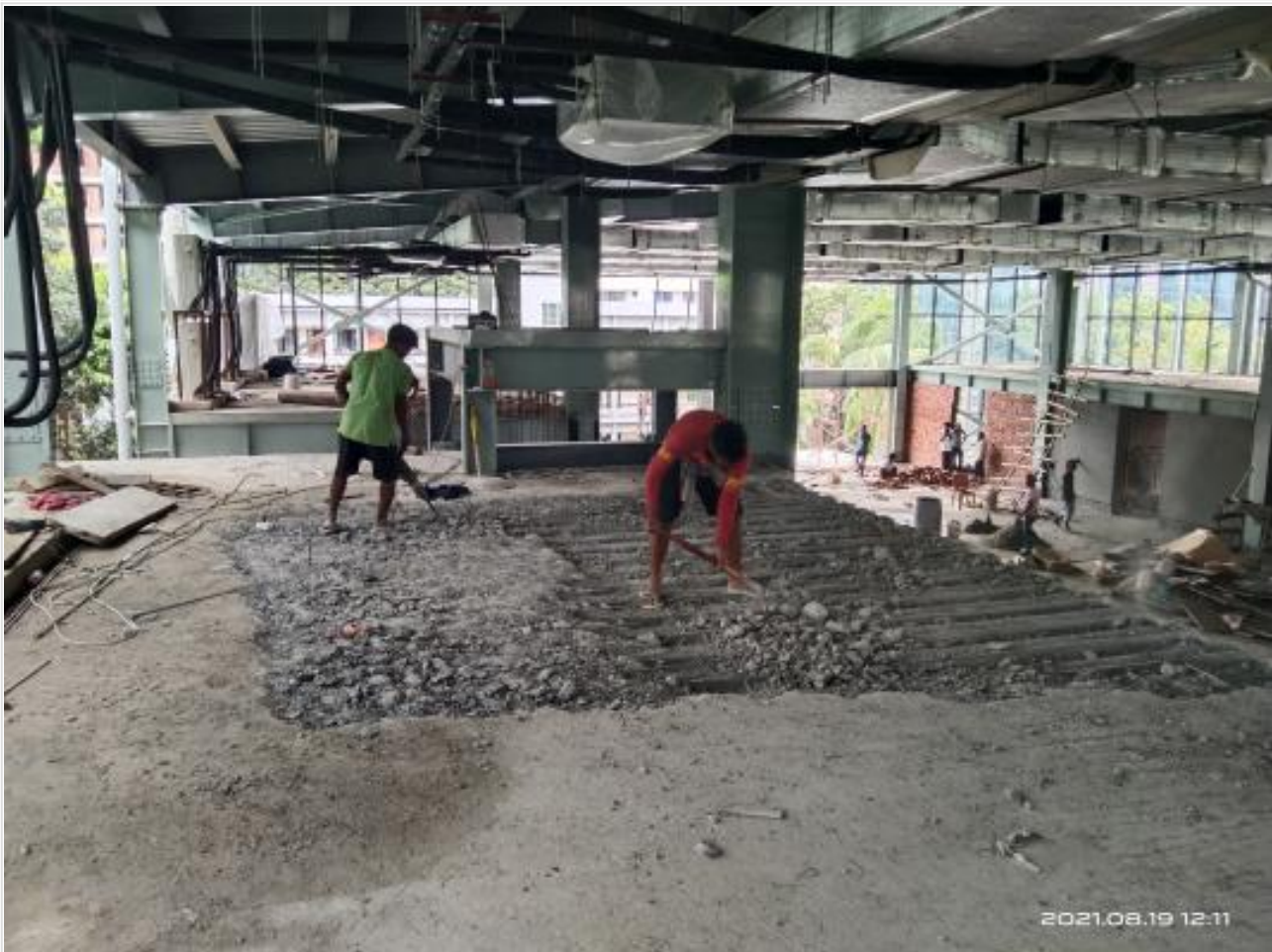
FF Mezzanine floor dismantling on 19-08-21
