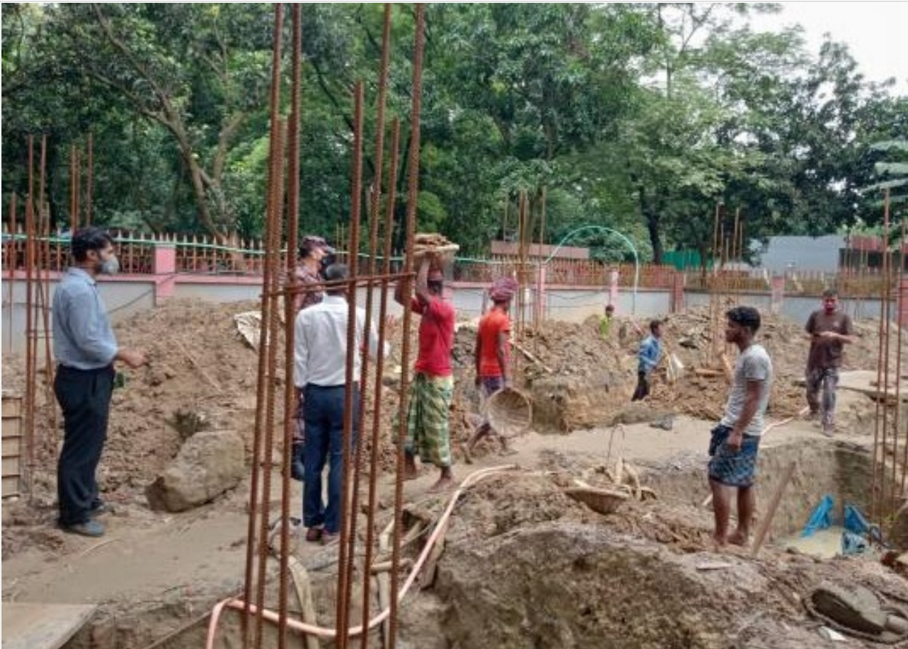
Sub-station grade beam earth cutting wor on 02-08-21
