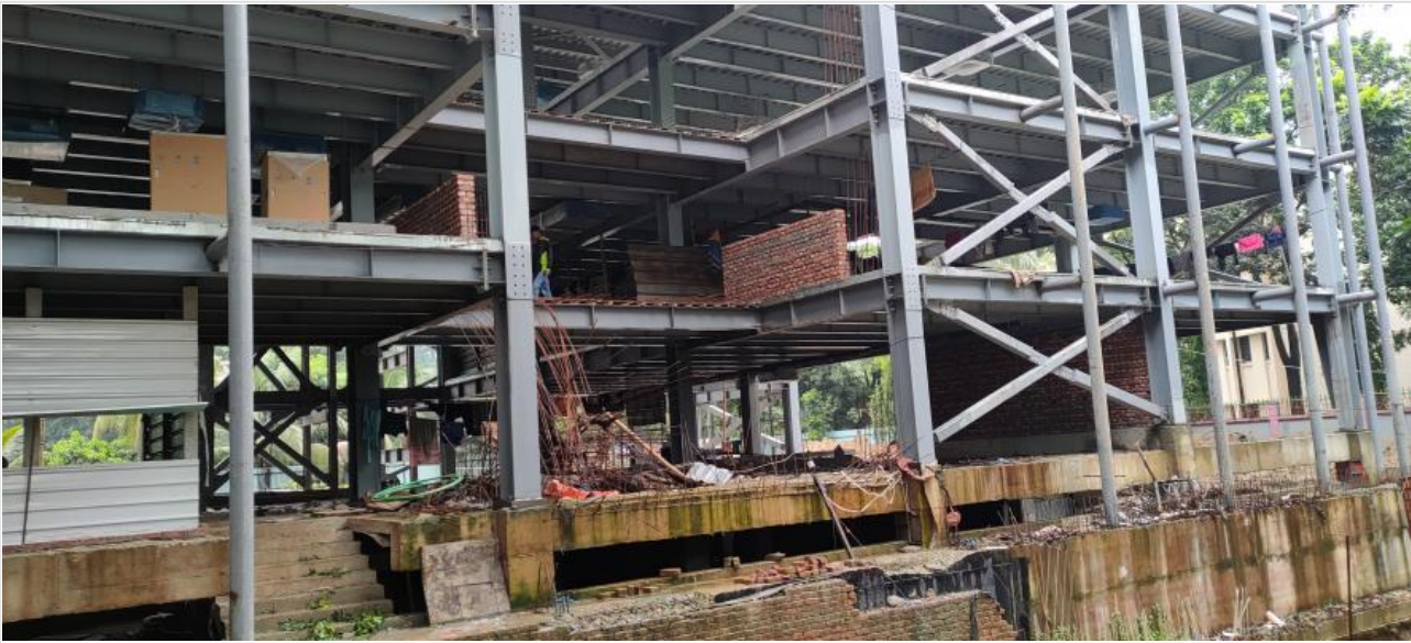
Gr.Floor Mezzanine Brick Work on 16-06-21
