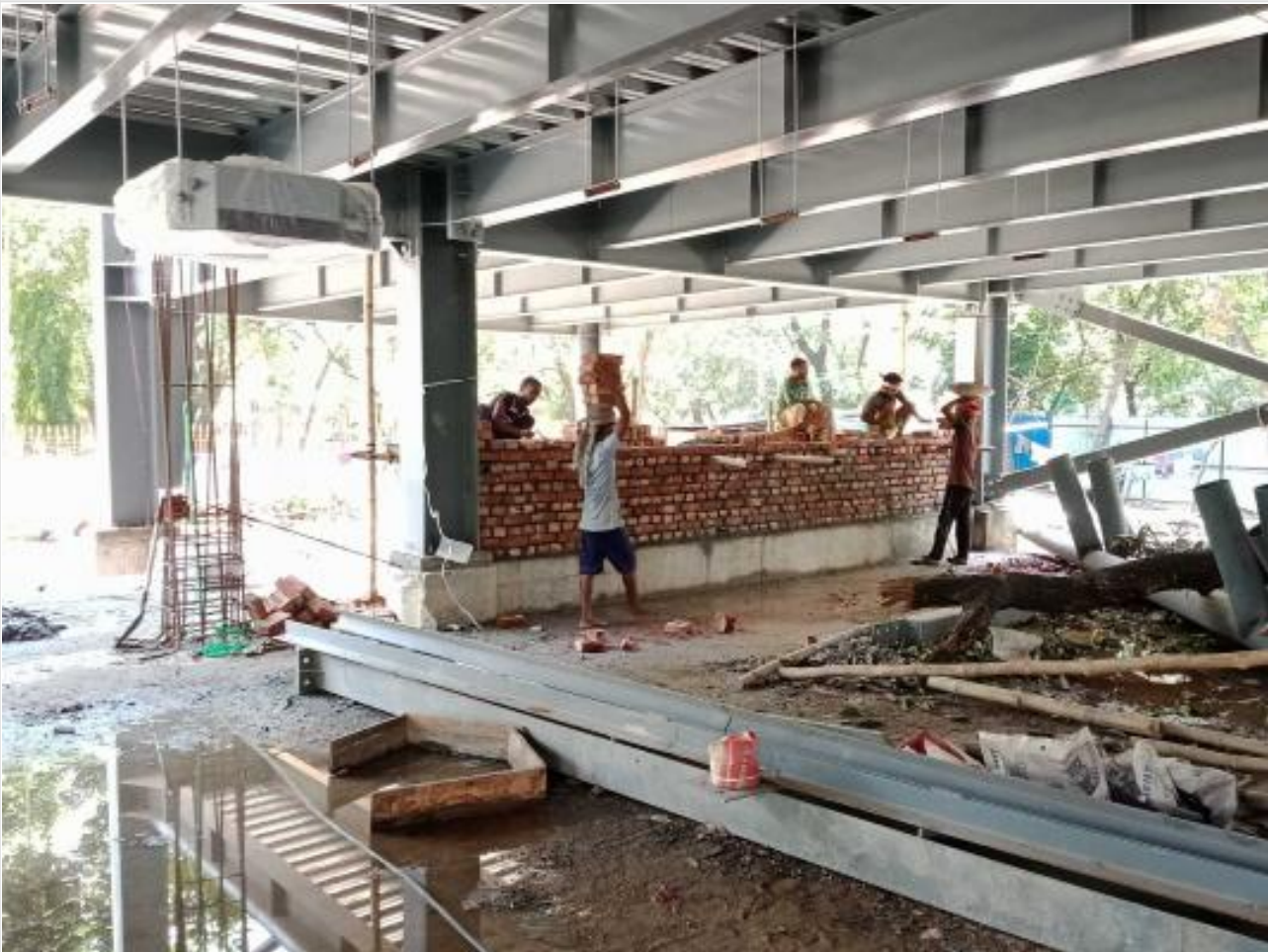
Ground Floor Brick Work on 22-05-21
