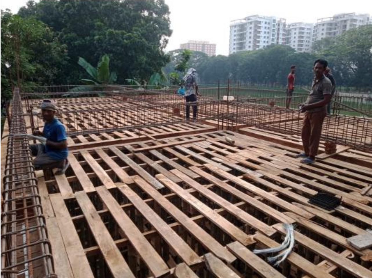
Generator room slab shuttering on 26-09-21
