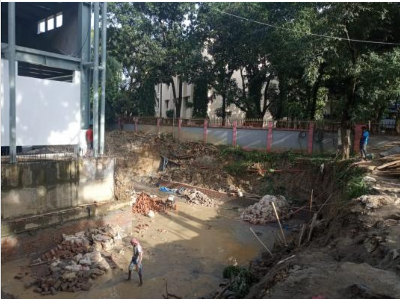
Earth remove from fire tank base on 22-09-21
