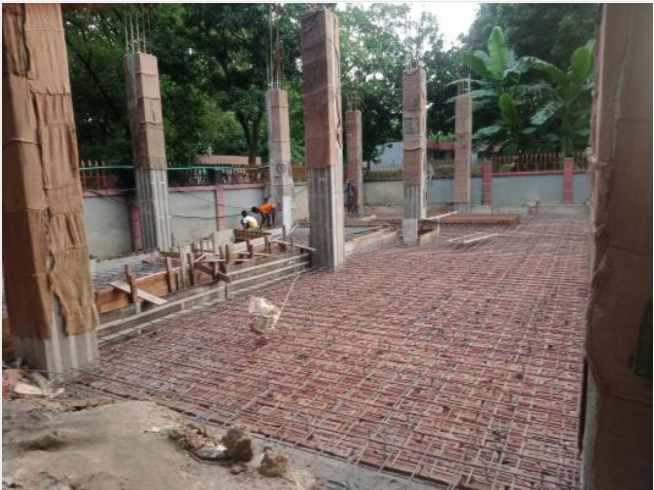
Generator room floor rod binding on 06-09-21
