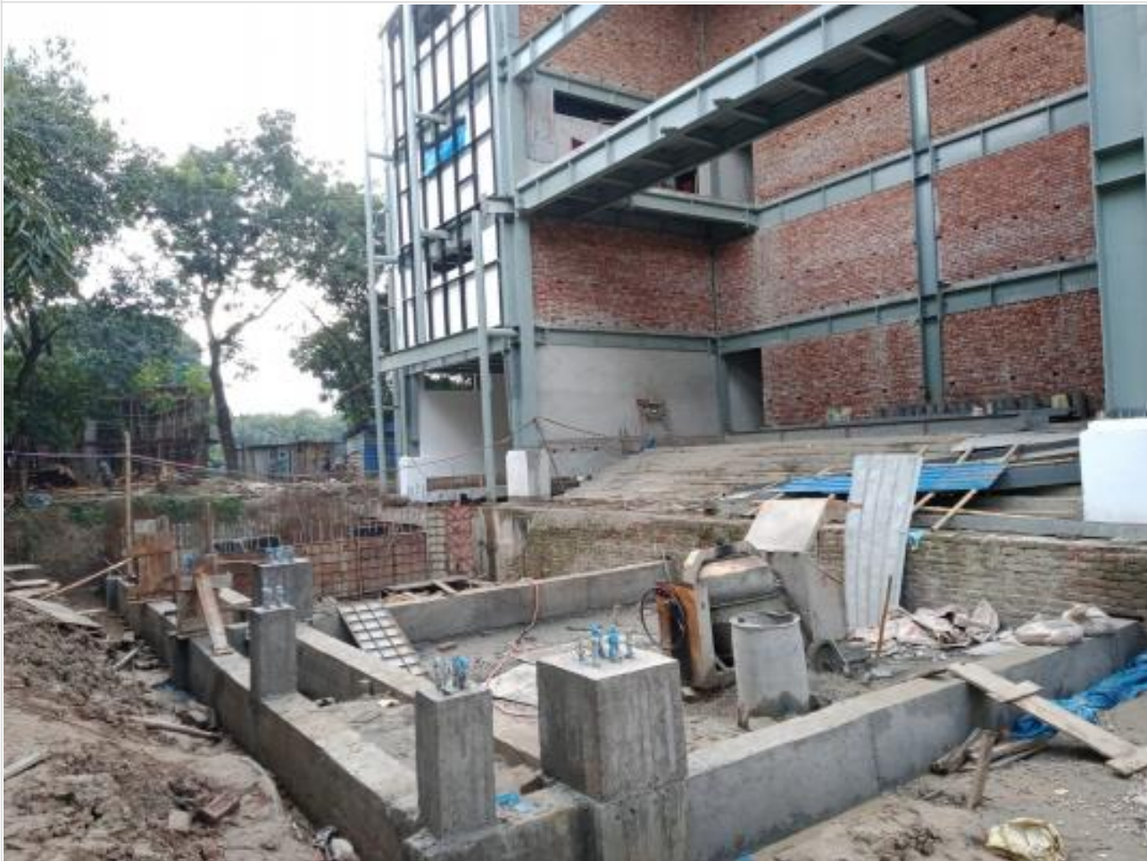
Canopy short column and GB casting on 18-10-21
