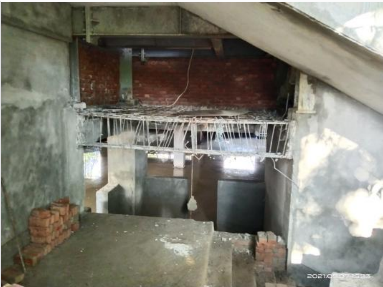
Beam dismantling for MDB Room on 07-09-21
