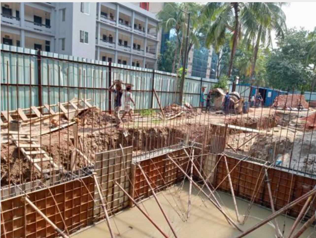
Domestic Water Tank-1st Lift Concreting on 04-06-21
