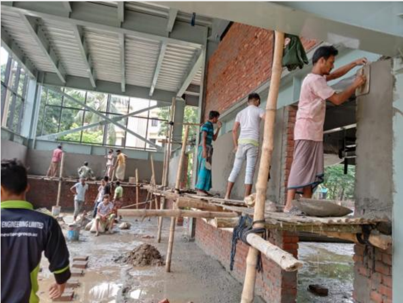
GF Mezzanine Shear Wall Plasteing on 09-08-21
