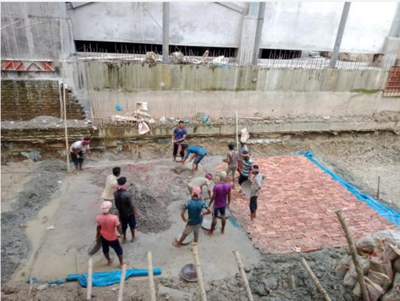
Fire tank base cc casting on 11-09-21
