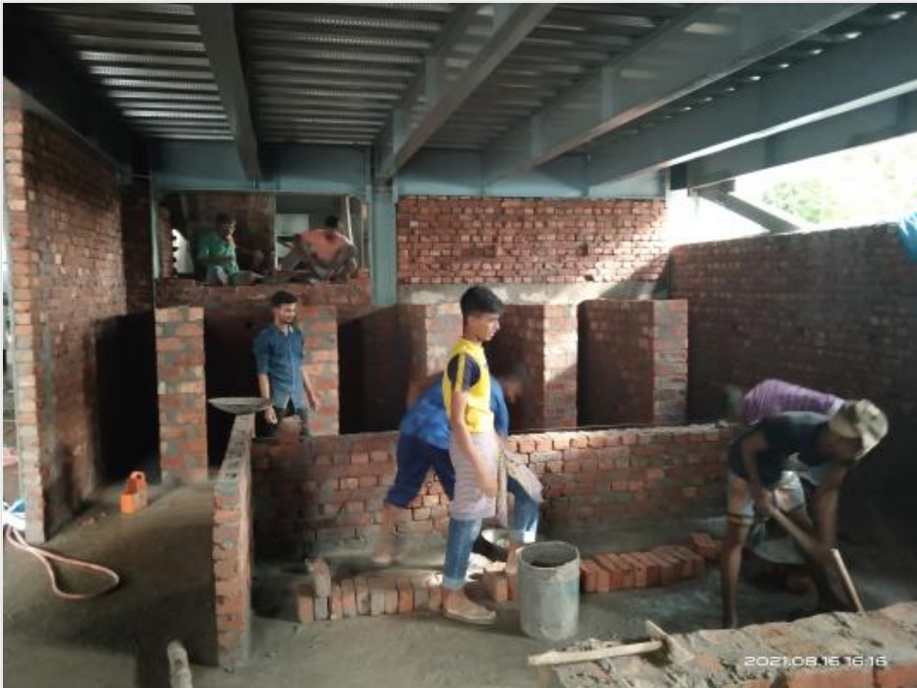
GF Brick work on 16-08-21
