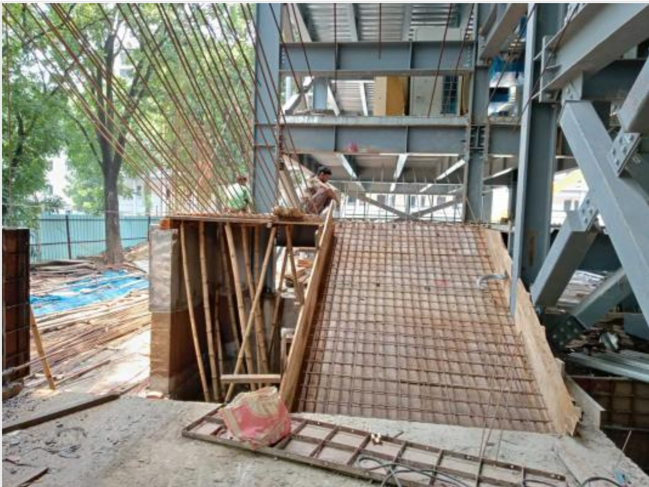
Ground Floor Stair Shuttering on 05-06-21
