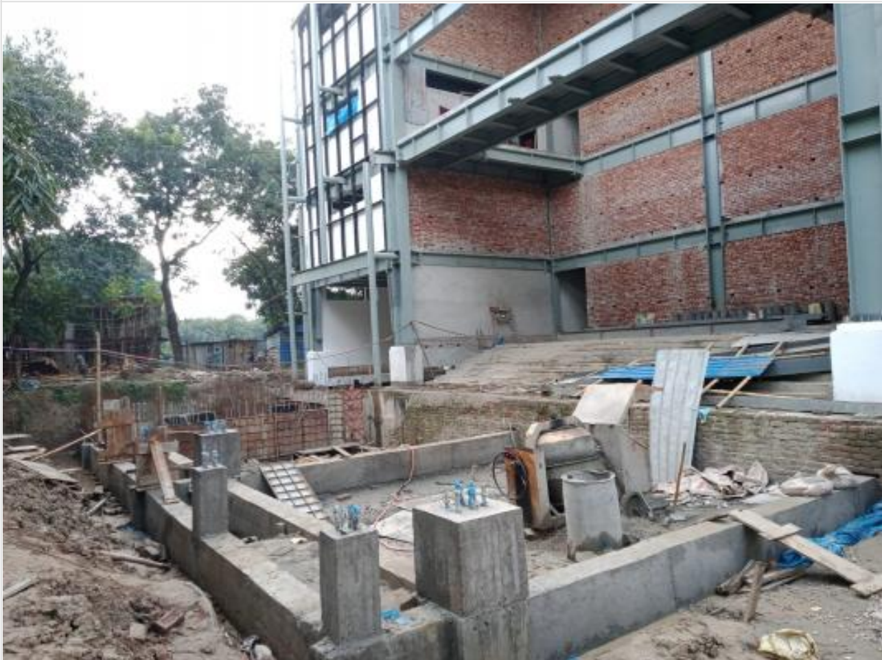
Canopy short column and GB casting on 18-10-21
