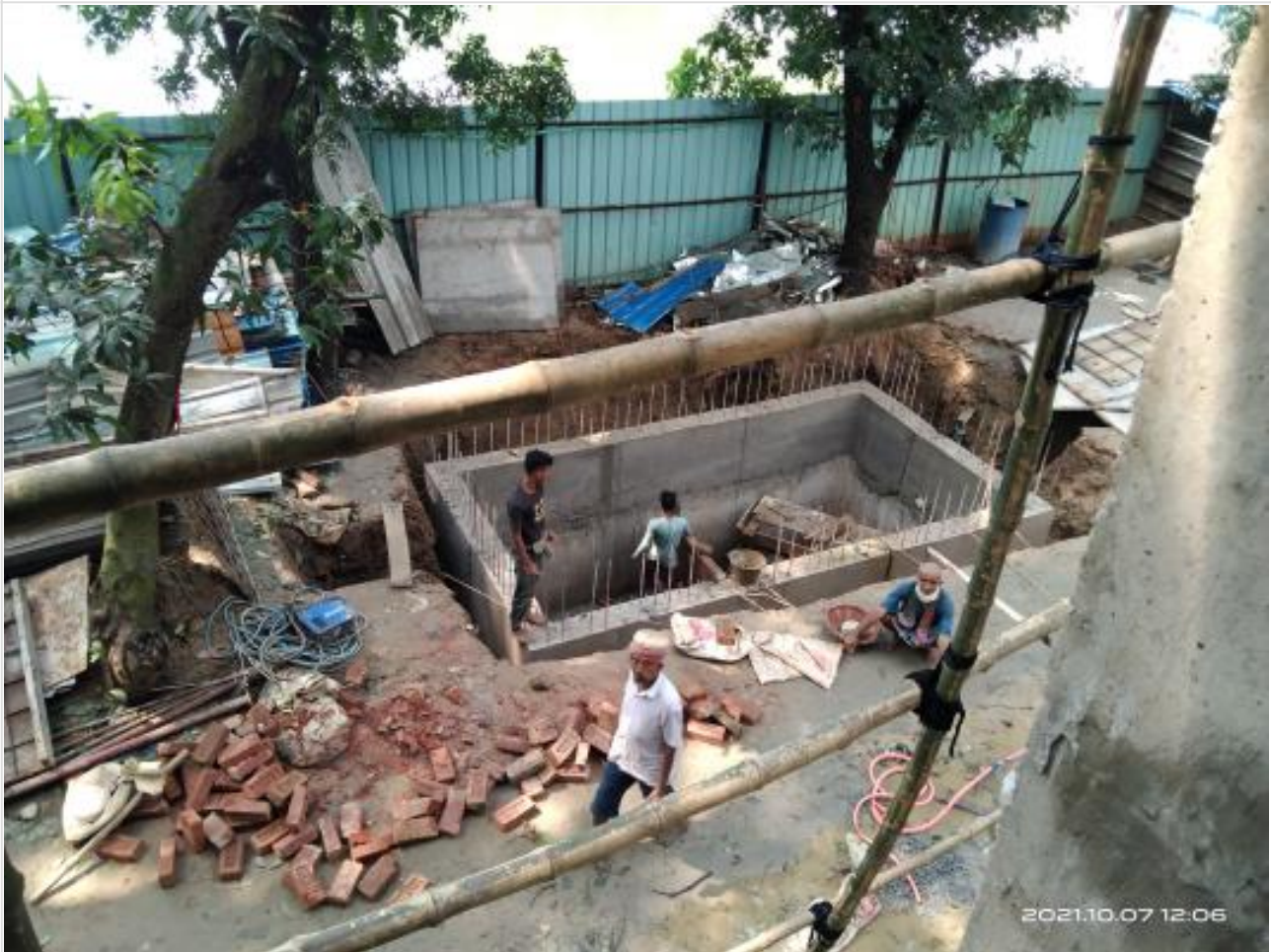
Septic partition wall on 07-10-21
