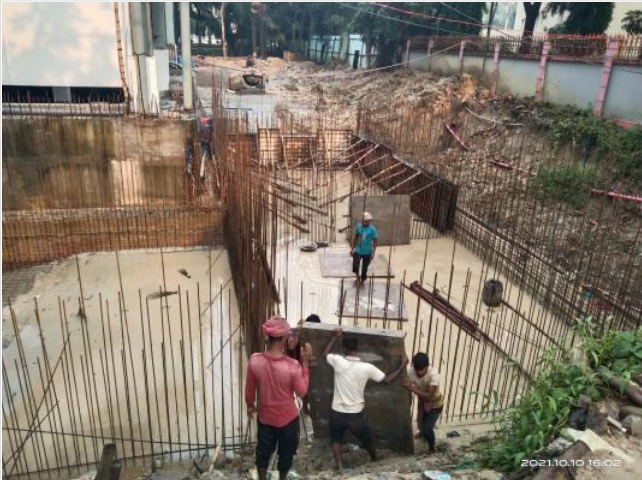
Fire tank wall shuttering and tasing on 10-10-21
