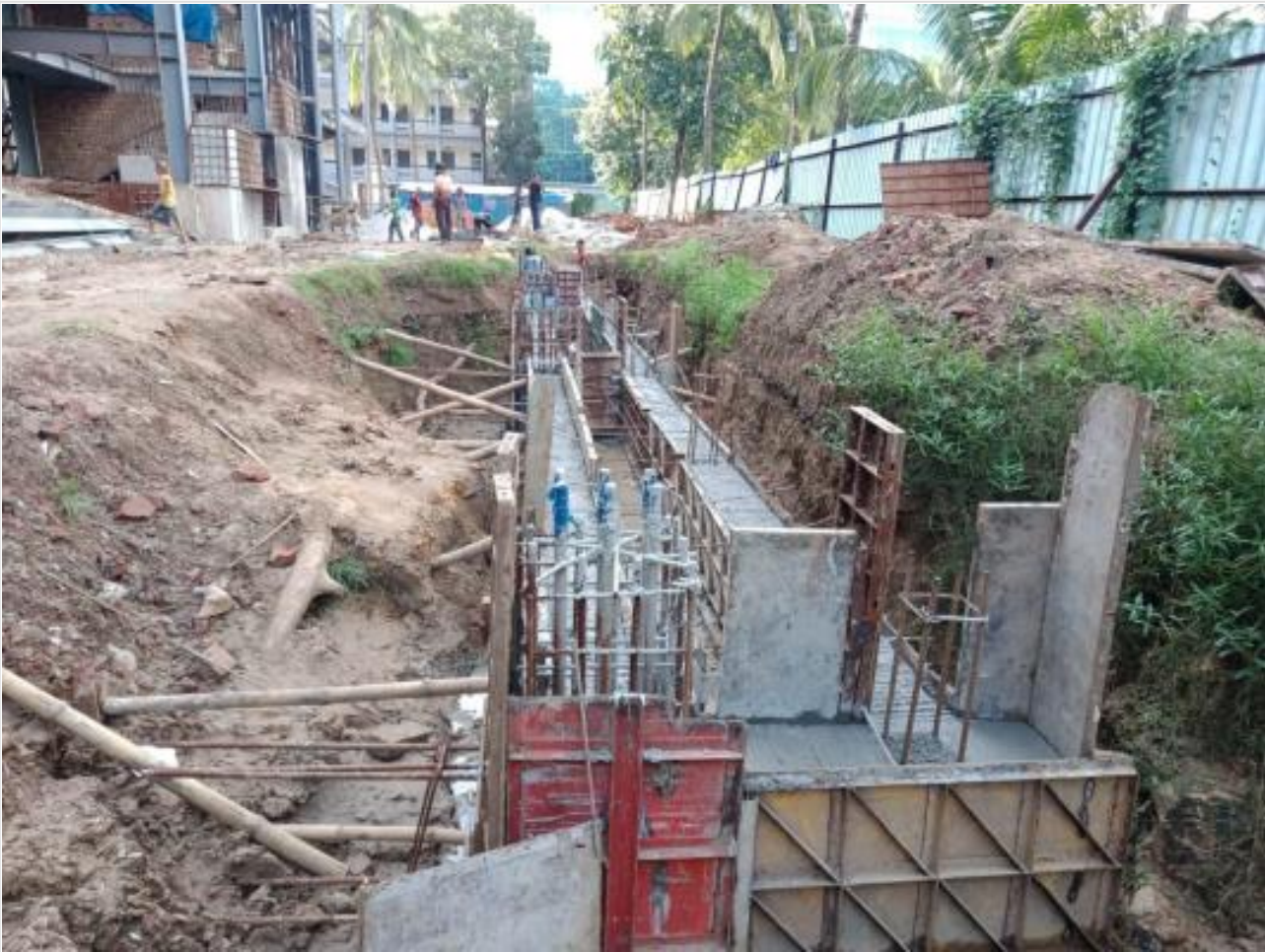
Porch Grade Beam Concreting on 25-06-21
