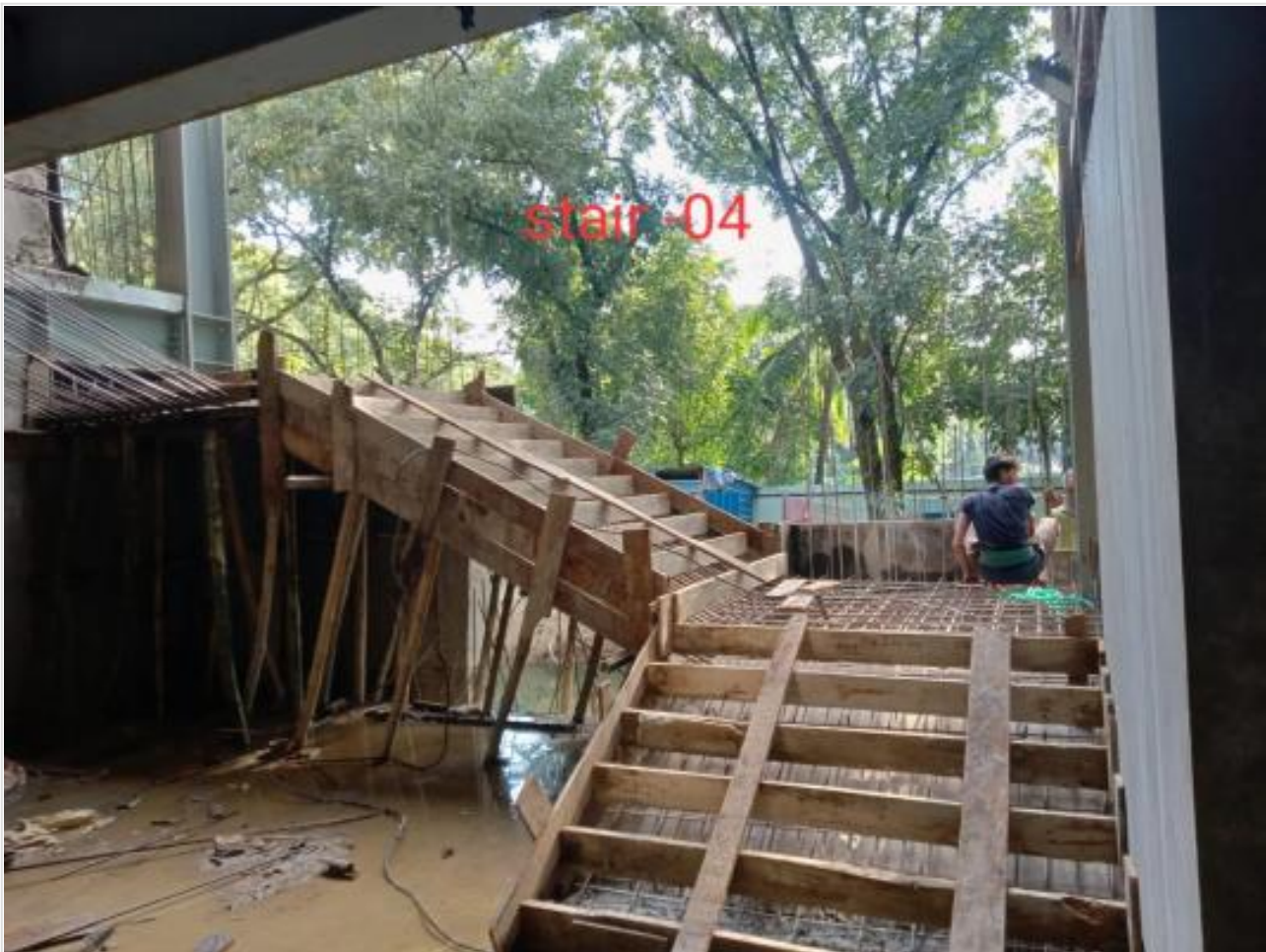
GF Stair casting on 31-08-21
