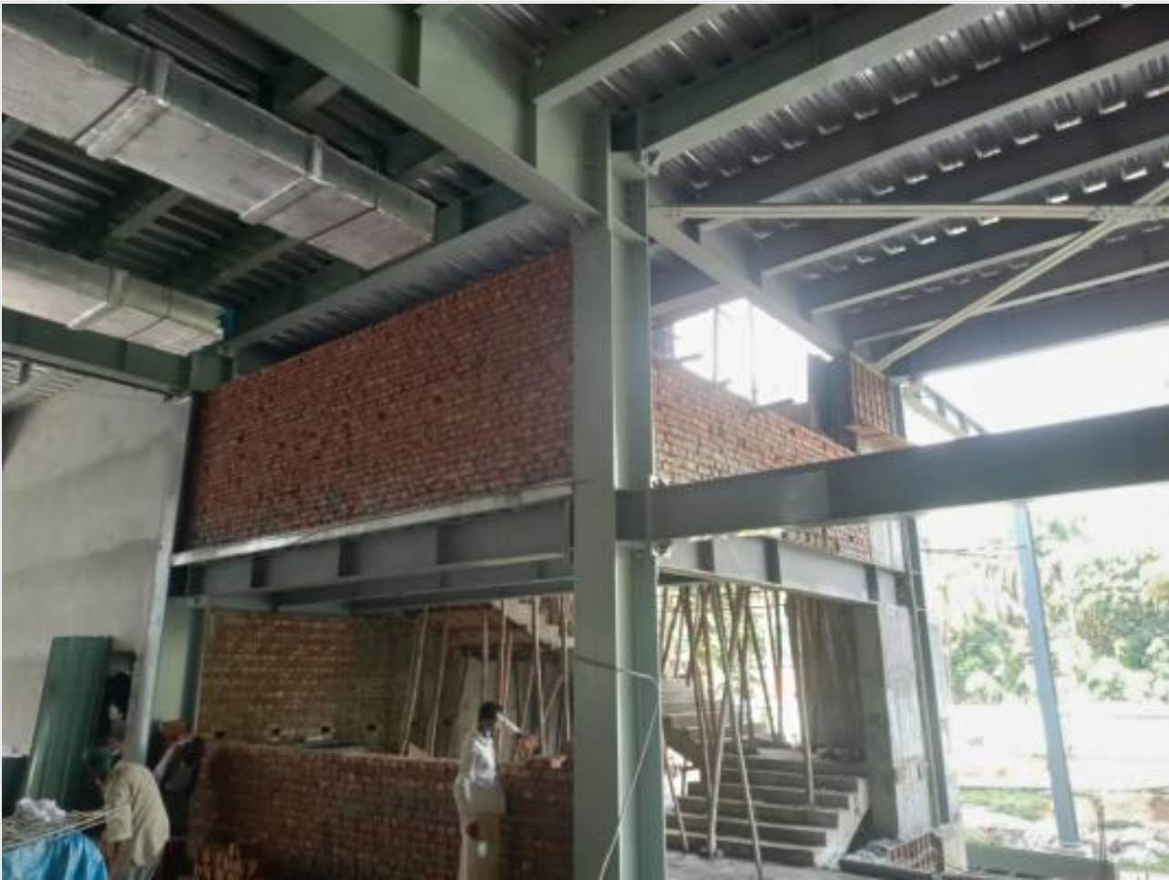
GF Mezzanine brick work on 05-08-21
