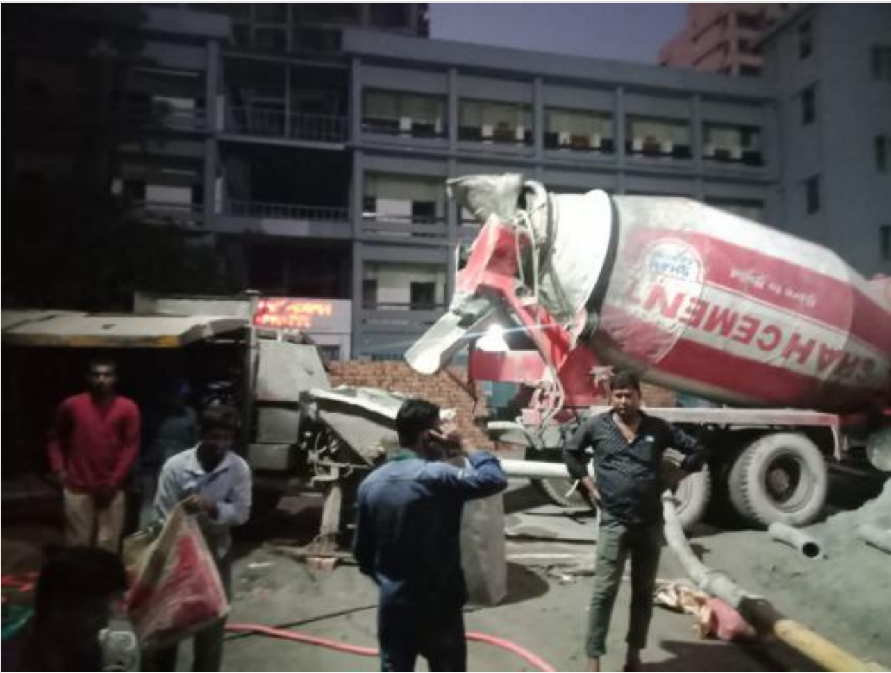
RMC Truck for Fire Tank and Porch Slab C on 16-11-21
