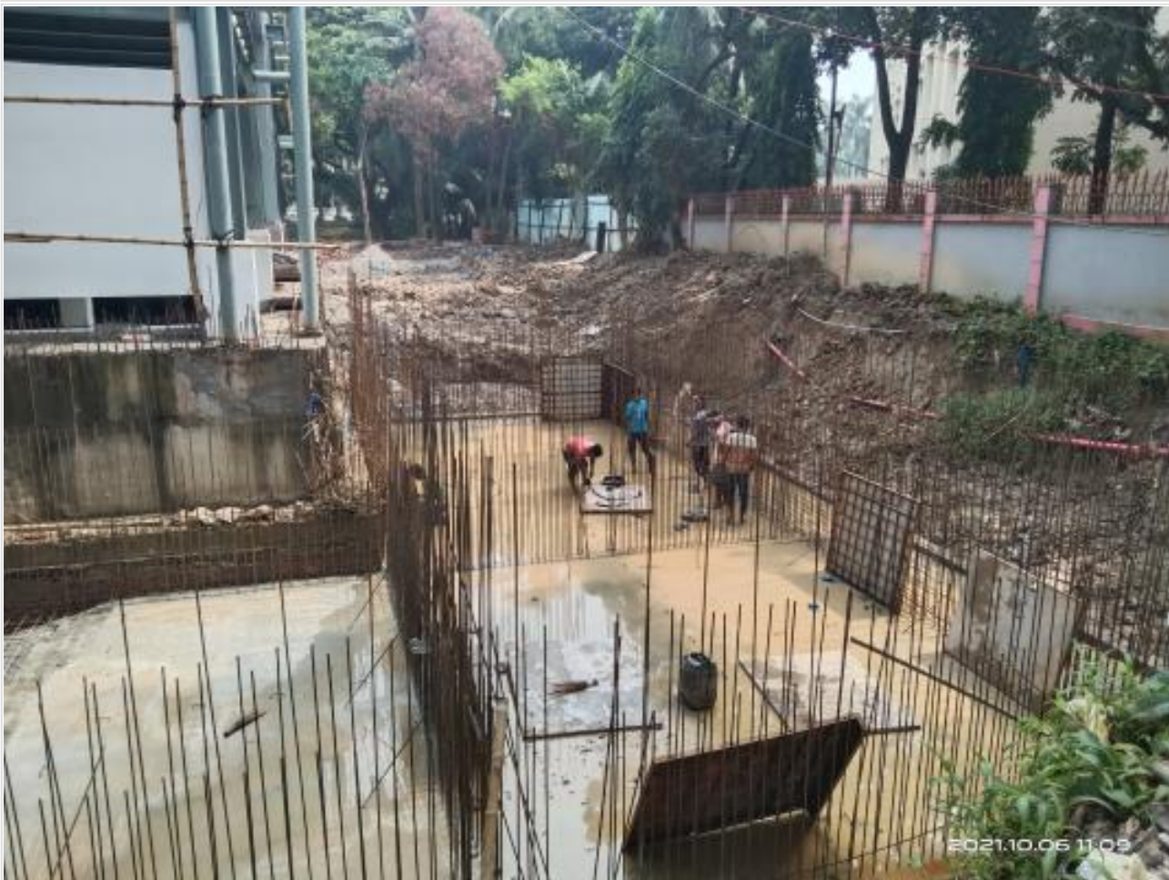
Fire tank wall shuttering on 06-10-21
