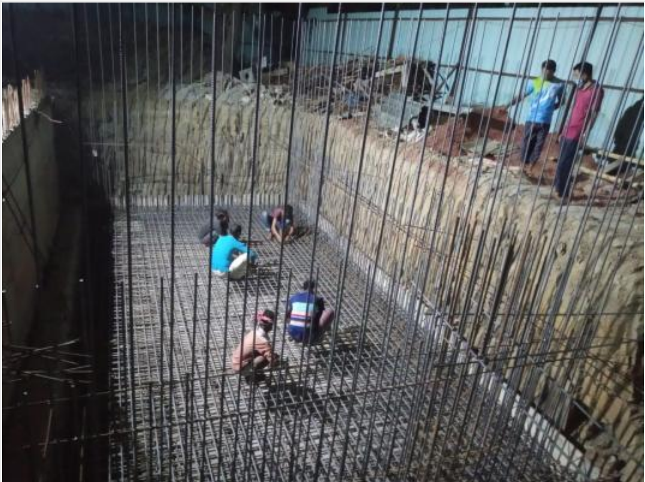
Domestic Water Tank Re-bar work on 01-05-21
