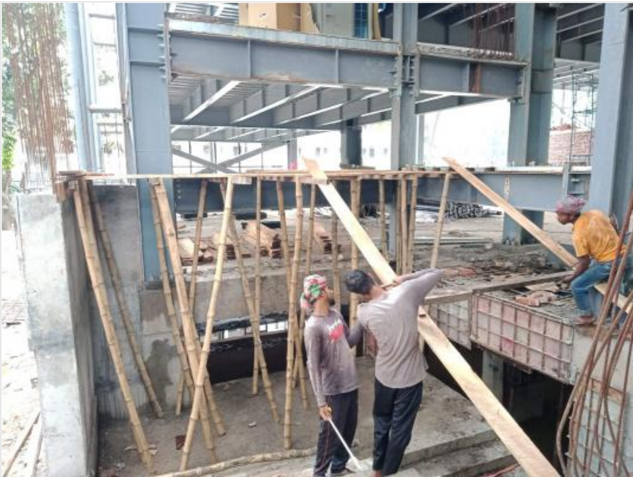
Ground Floor-Stair Shuttering on 04-06-21
