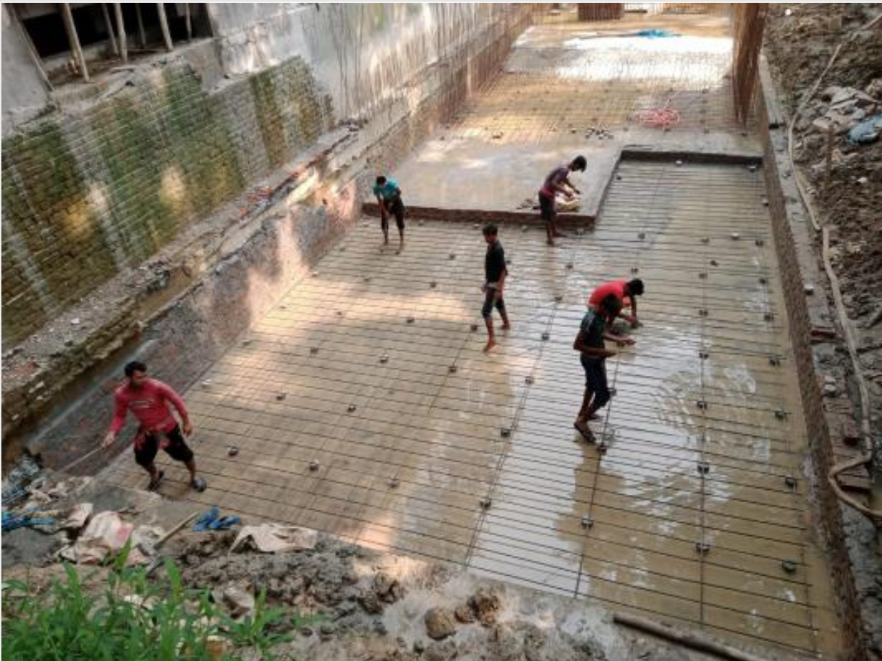
Fire tank base rod binding on 12-10-21
