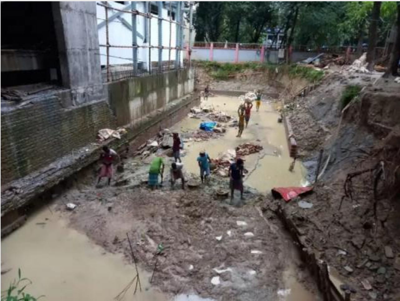
Fire tank base clean on 25-09-21
