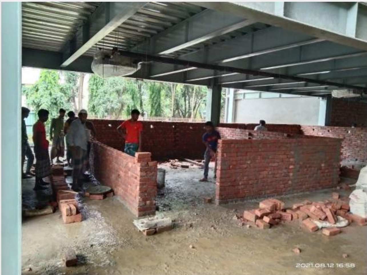
GF Brick work on 12-08-21
