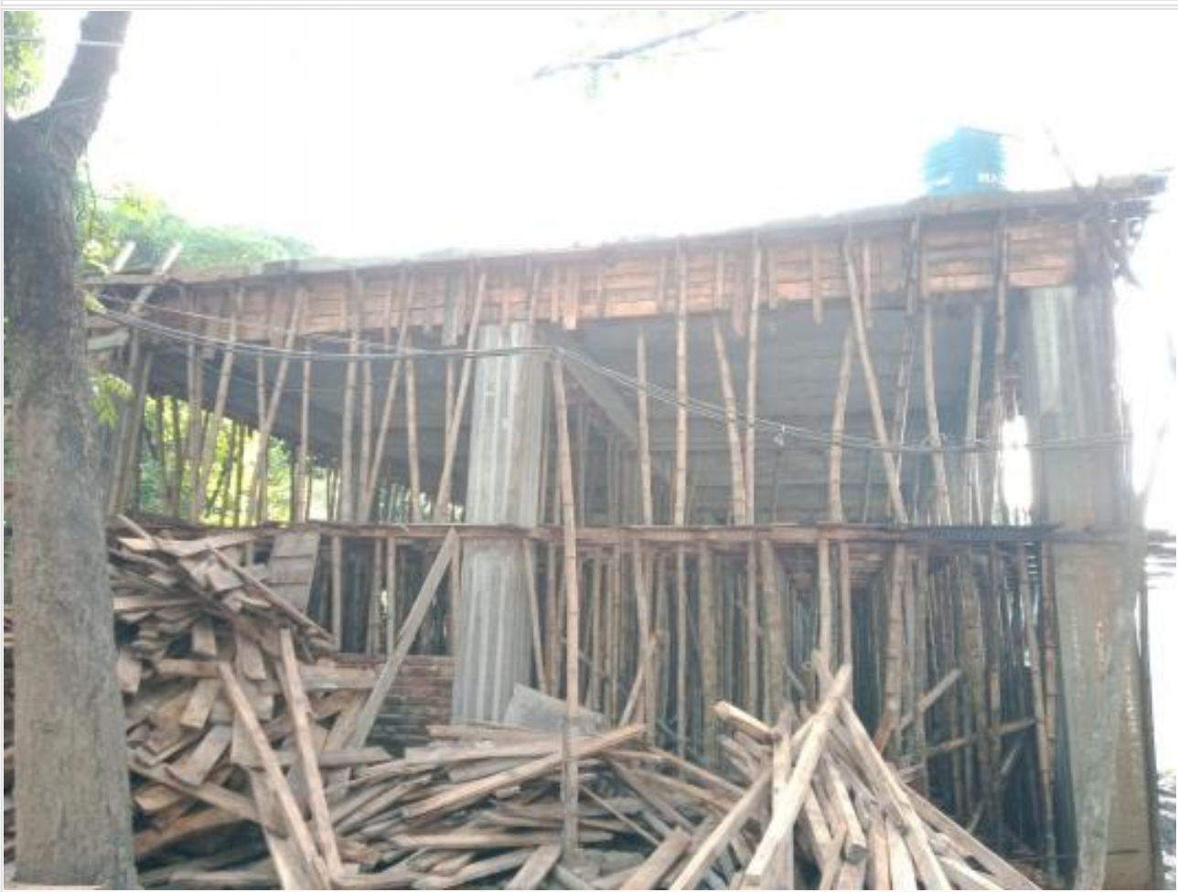
Generator room shutter remove on 16-10-21
