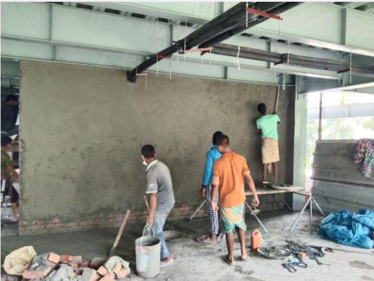
FF wall plaster on 22-08-21
