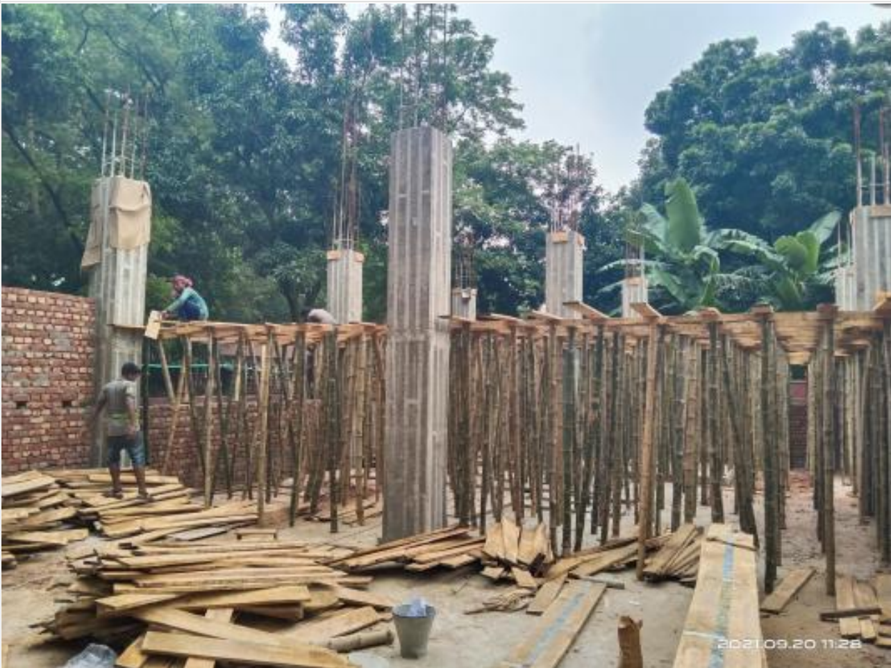
Sub-Station and Generator room staging f on 20-09-21
