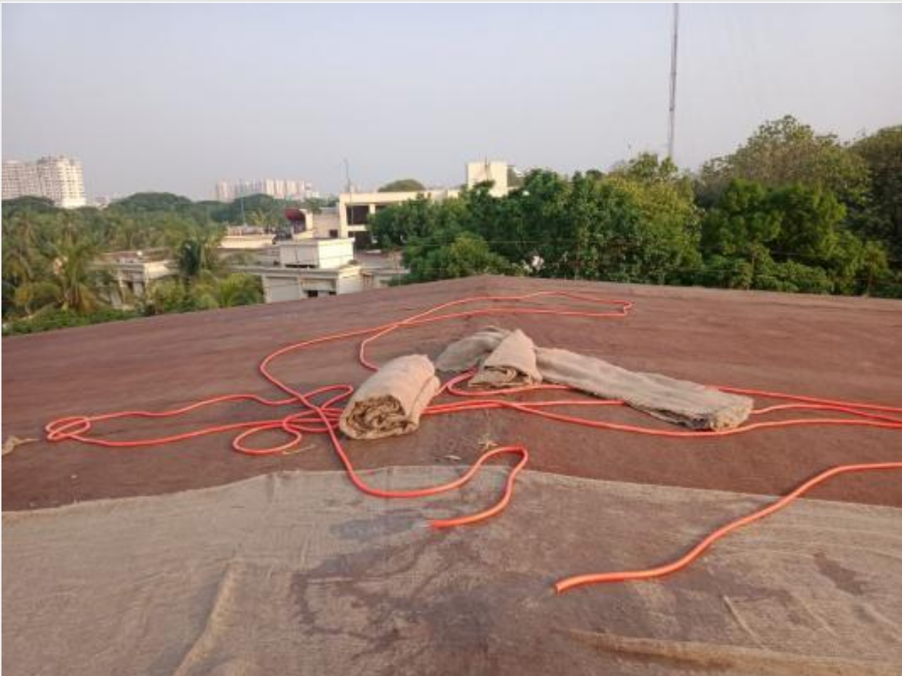
Hessian Cloth Covering after Concreting on 06-05-21
