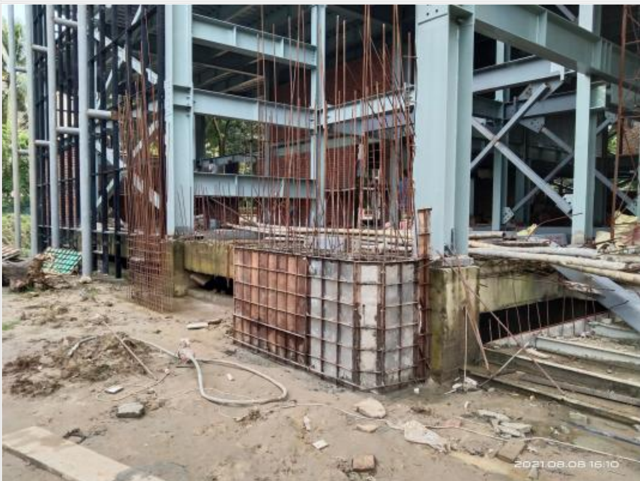
GF Stair no-3 shuttering and casting on 08-08-21
