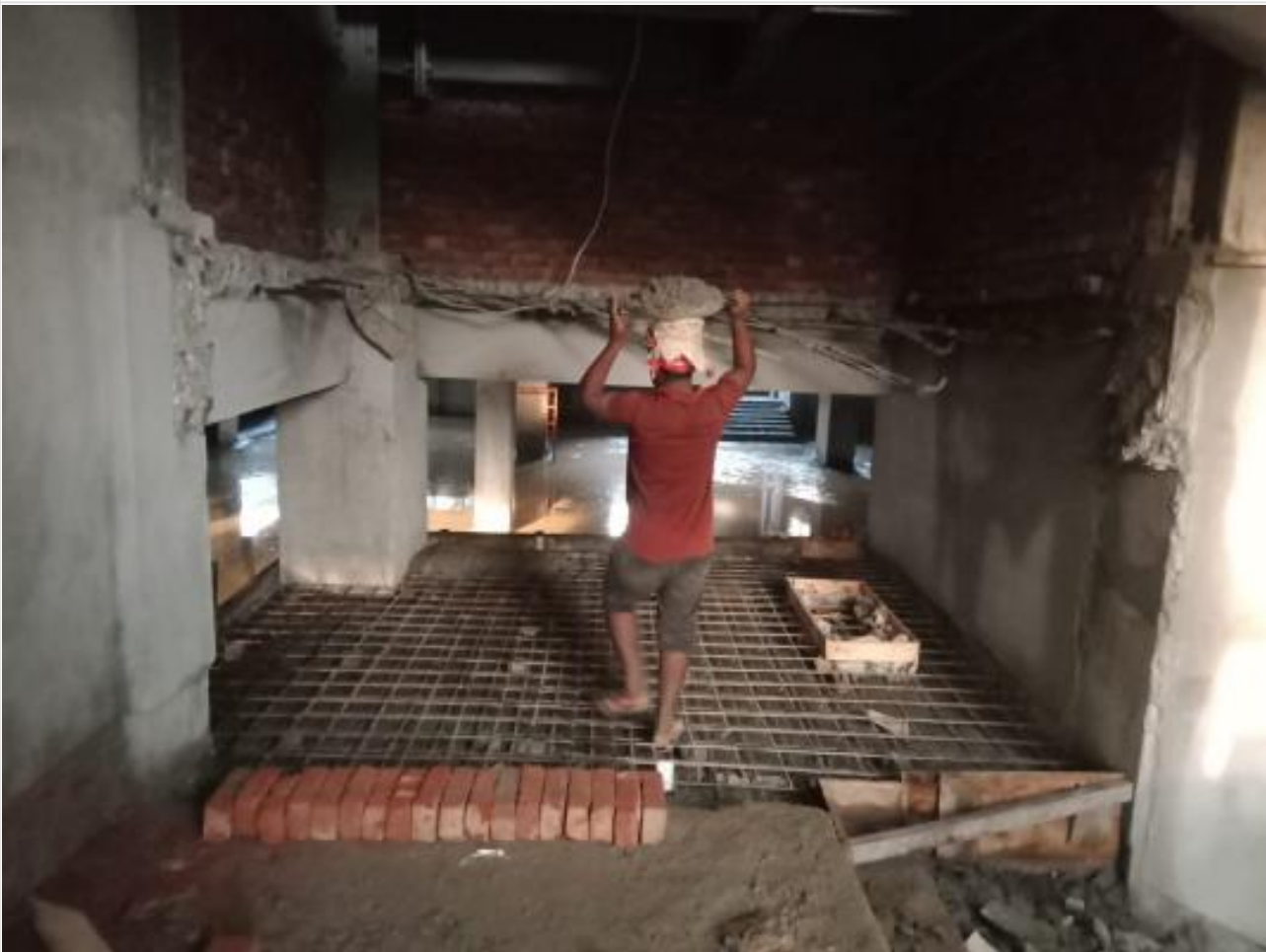
MDB room slab casting on 15-09-21
