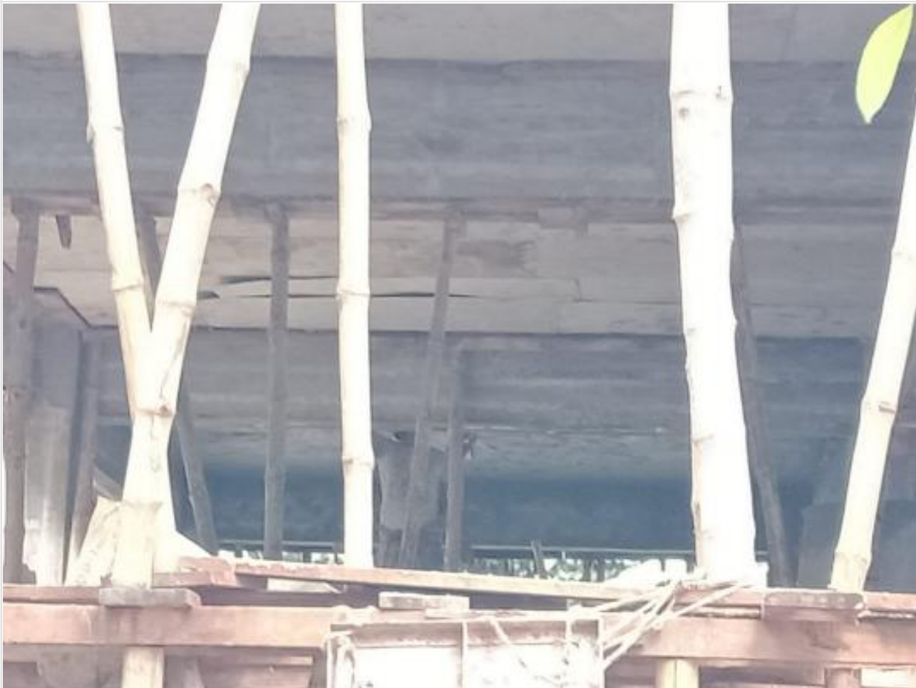
Generator Room shutter remove on 20-10-21
