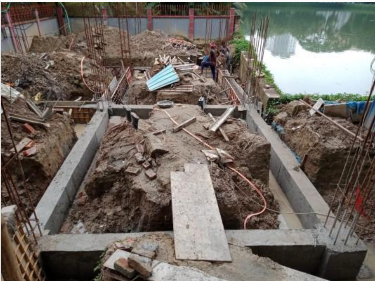
Substation Grade Beam Concreing on 09-08-21
