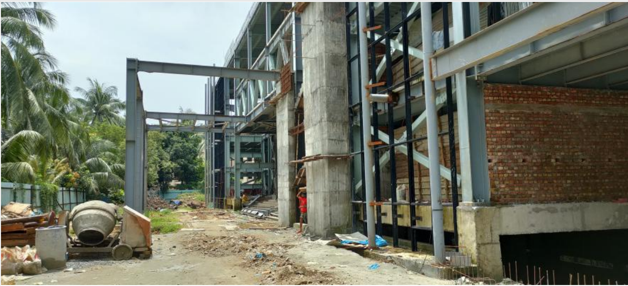
Steel Canopy Installing on 06-08-21
