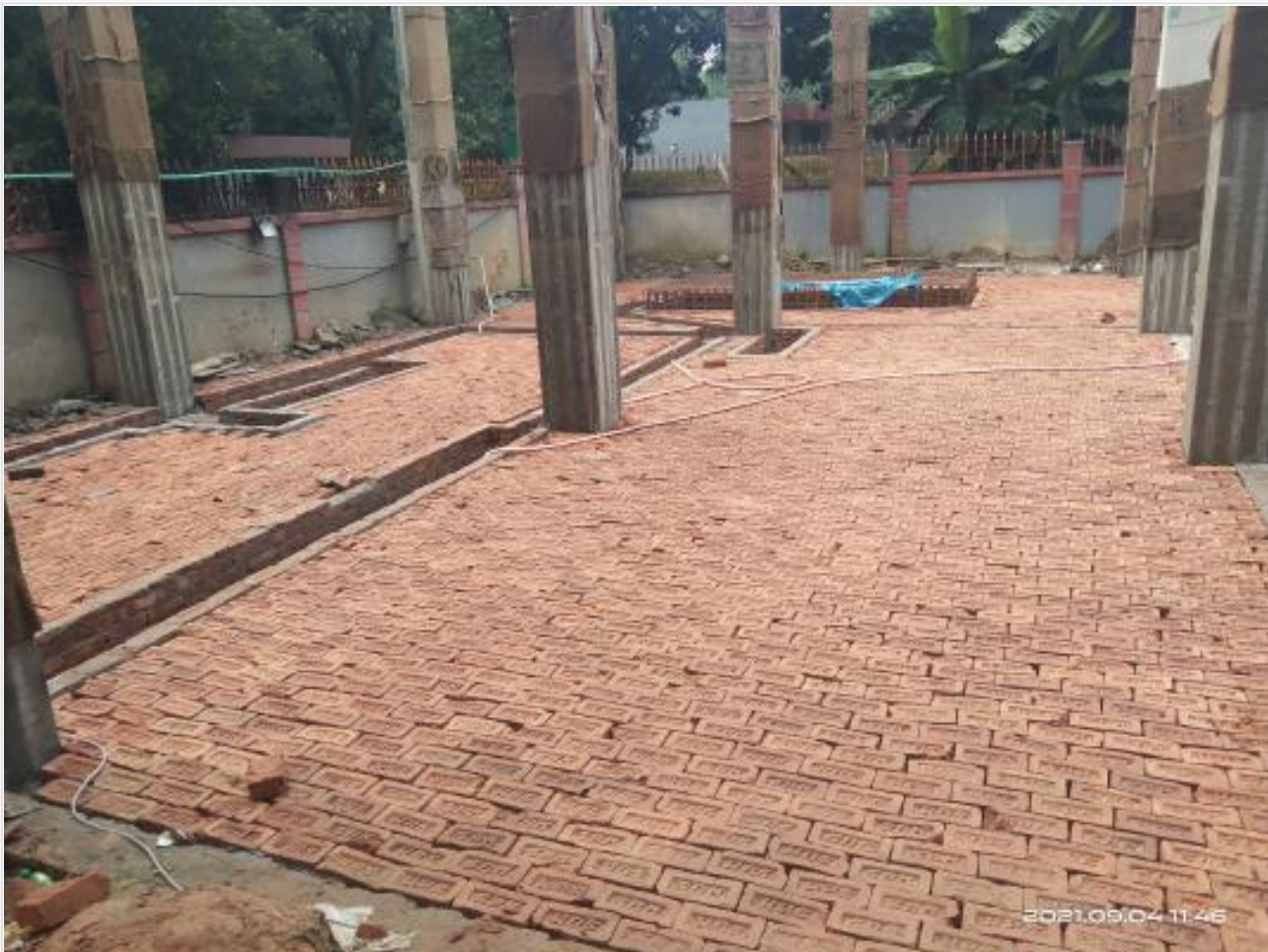
Generator room floor soling work on 04-09-21
