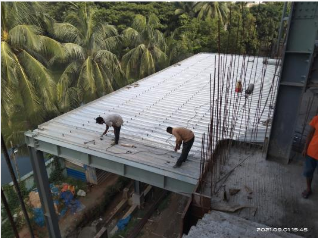
East Canopy Roofing work on 01-09-21
