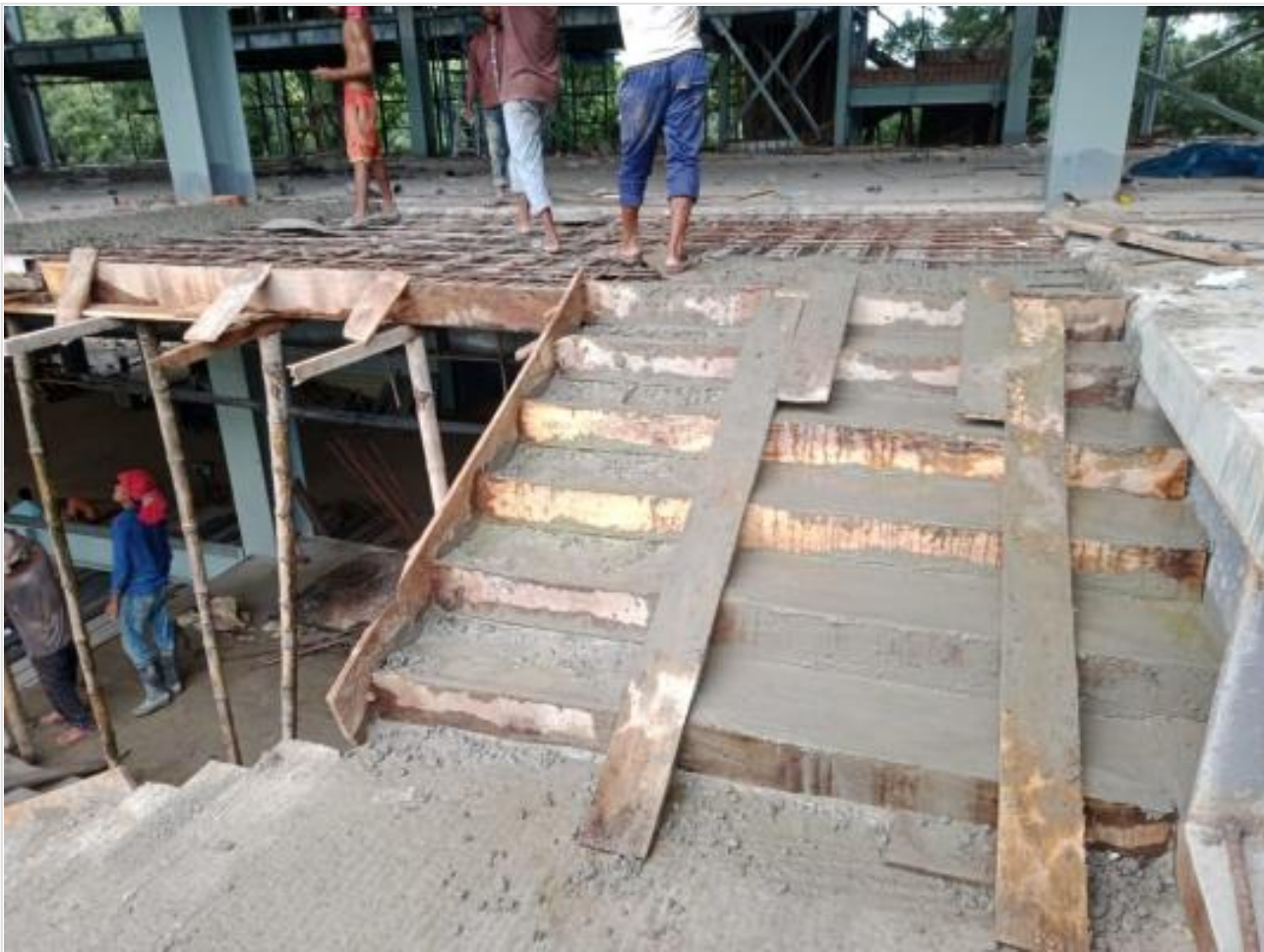
Gr.Floor Mezzanine Stair Concreting on 18-07-21
