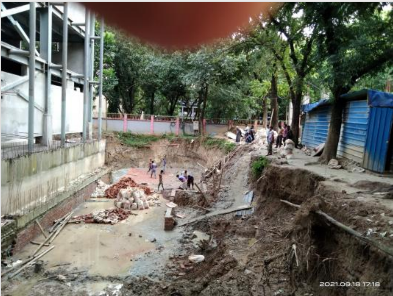
Fire tank cc work on 18-09-21
