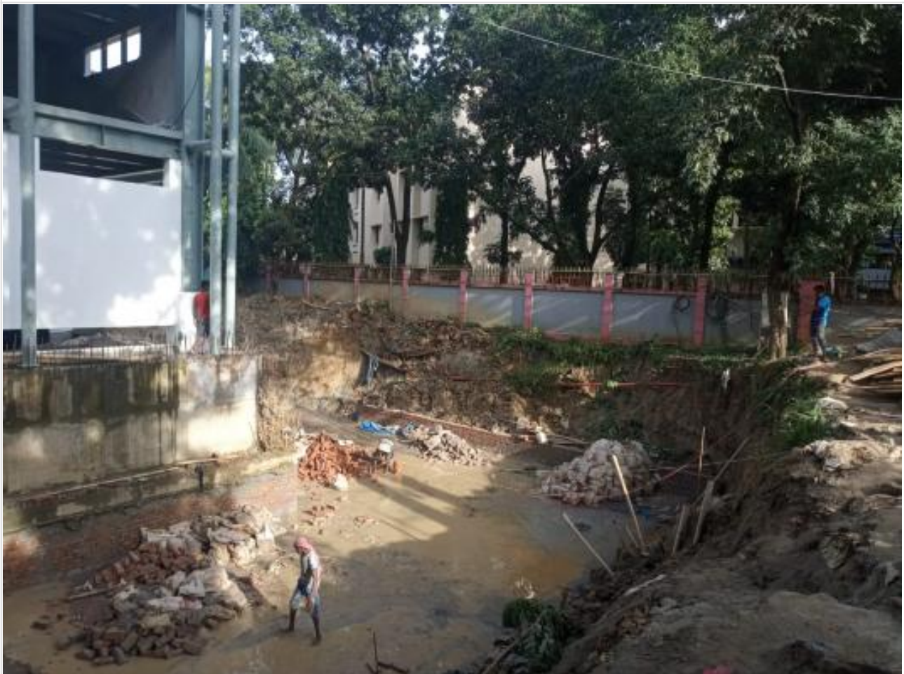
Earth remove from fire tank base on 22-09-21
