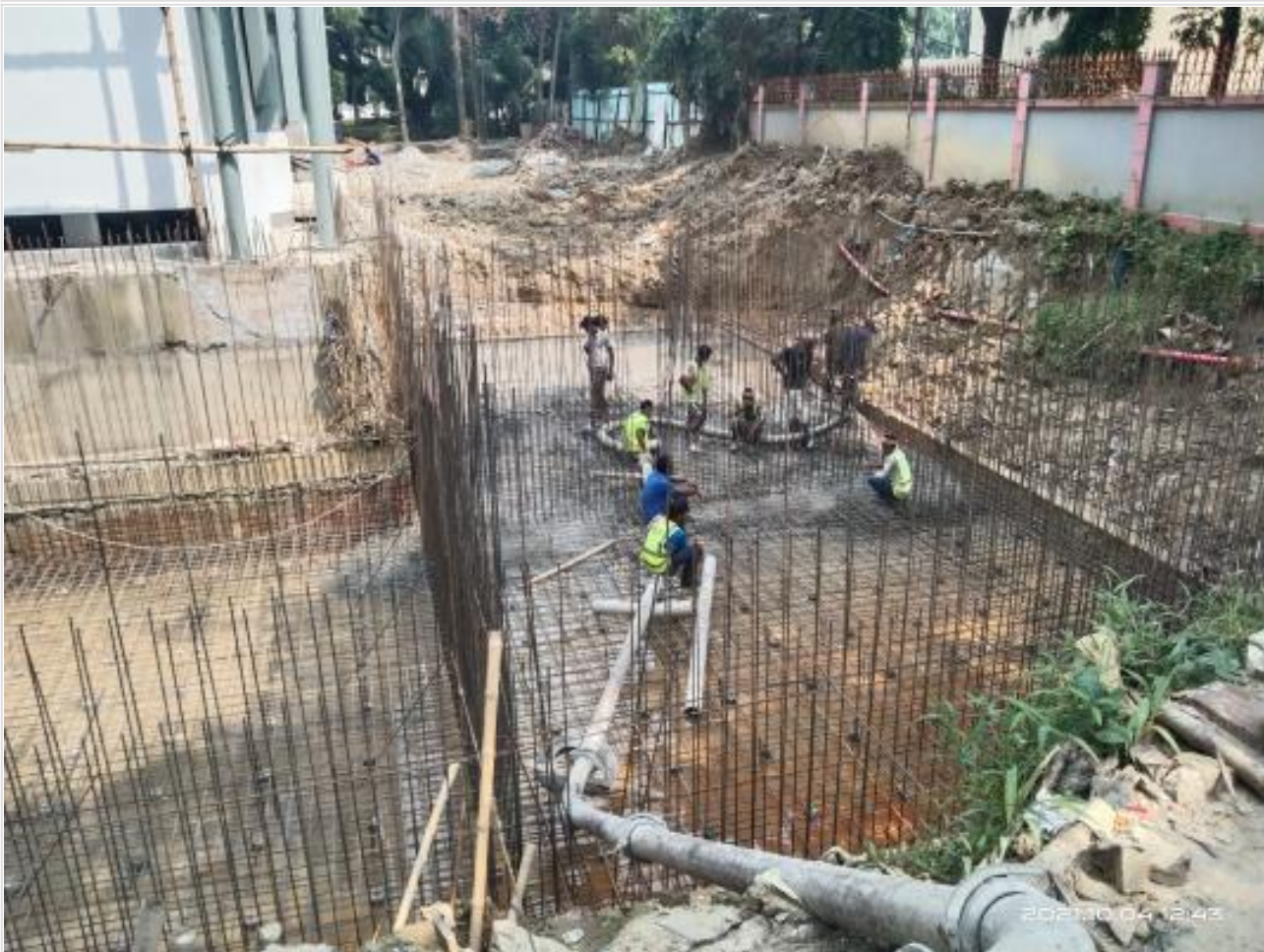
Fire tank base casting on 04-10-21
