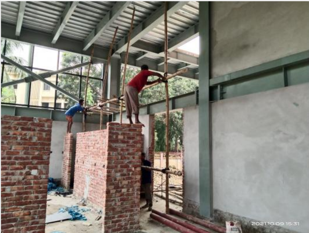
Scaffolding work for brick wall on 09-10-21
