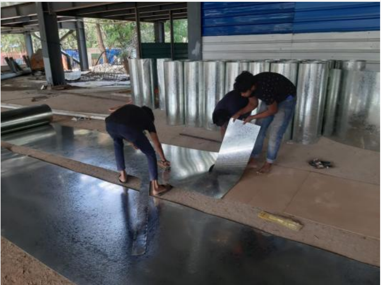
AC Duct Making on 09-05-21
