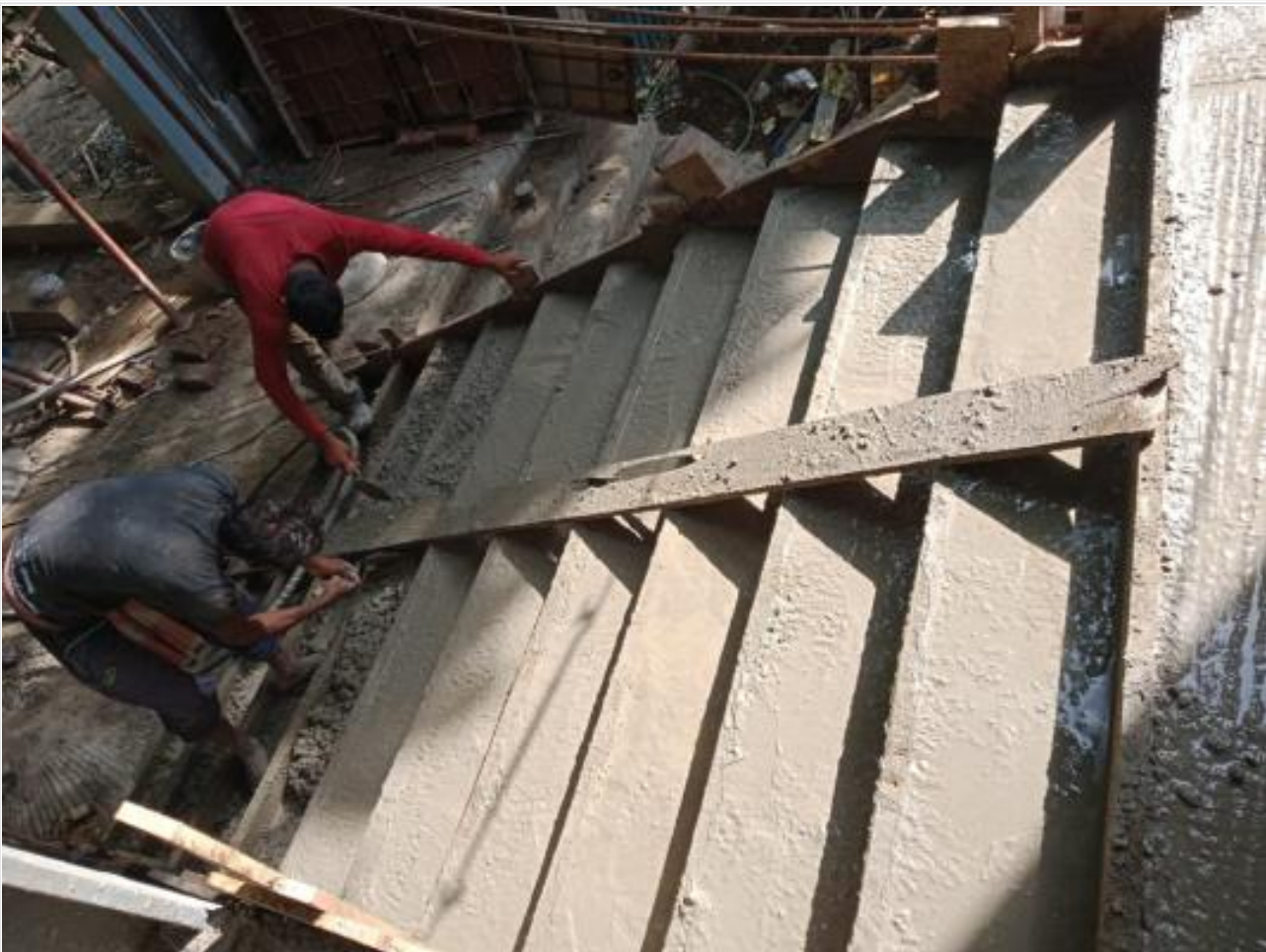
1st Floor Stair Concreting on 27-06-21
