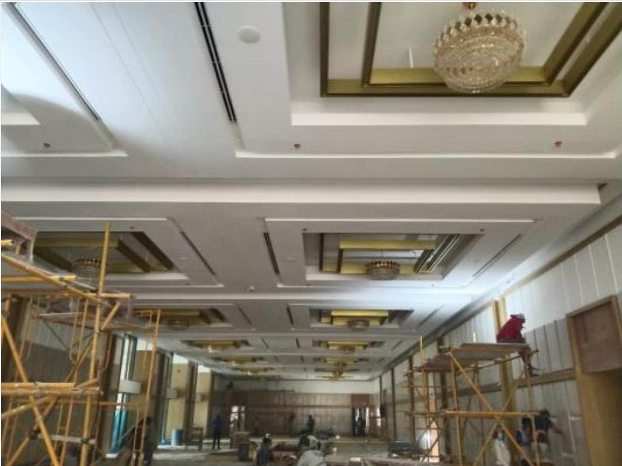
Ground Floor Interior Works on 12-12-21
