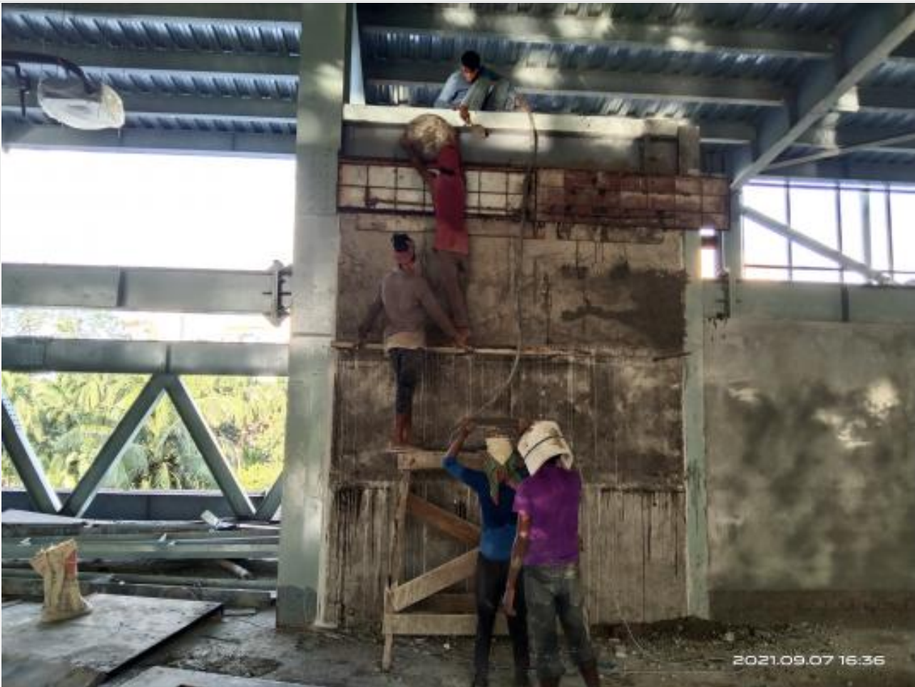
Lift wall casting on 07-09-21
