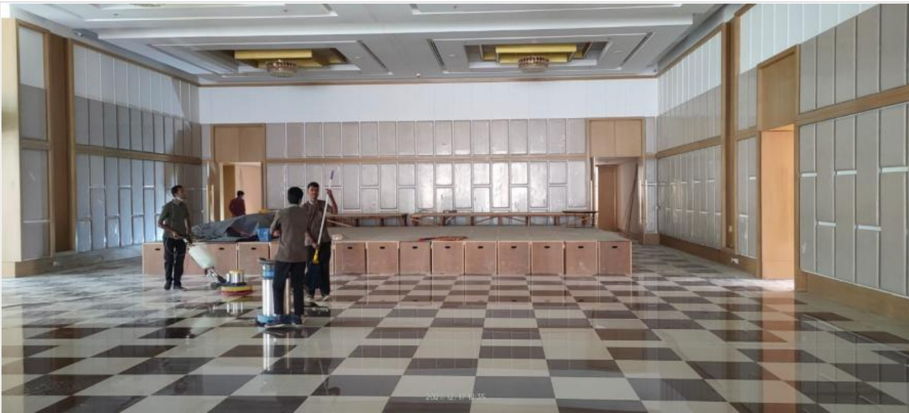
Stage work on 17-12-21
