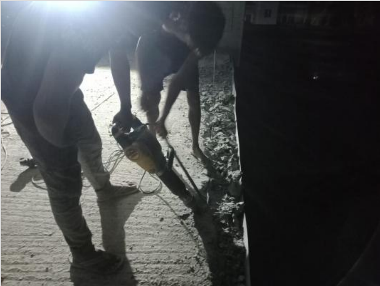
FF Mezzanine floor dismantling on 15-08-21
