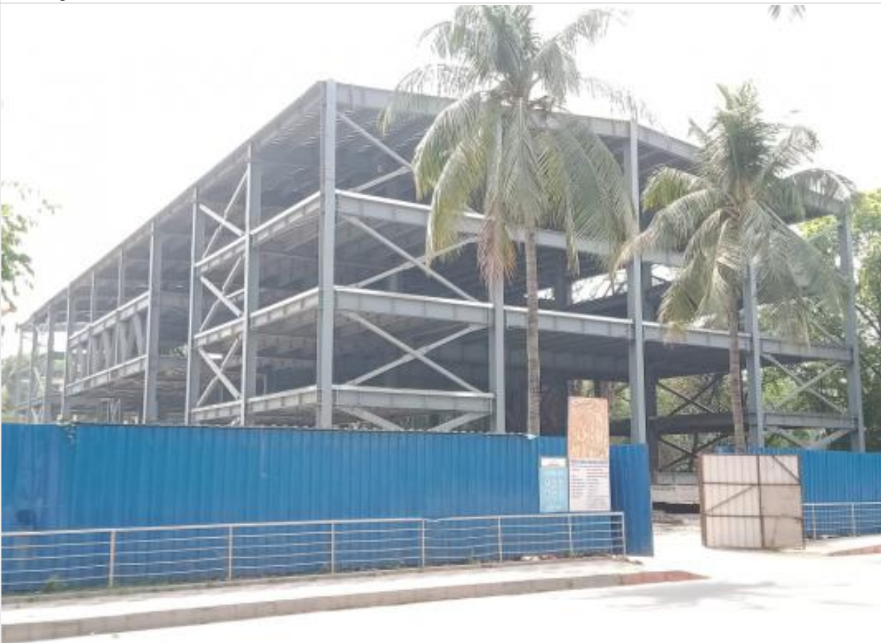
Decking Slab installation on 22-03-21
