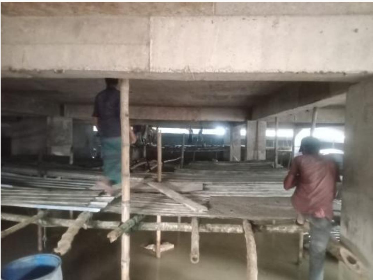
Basement Ceiling plaster on 03-09-21
