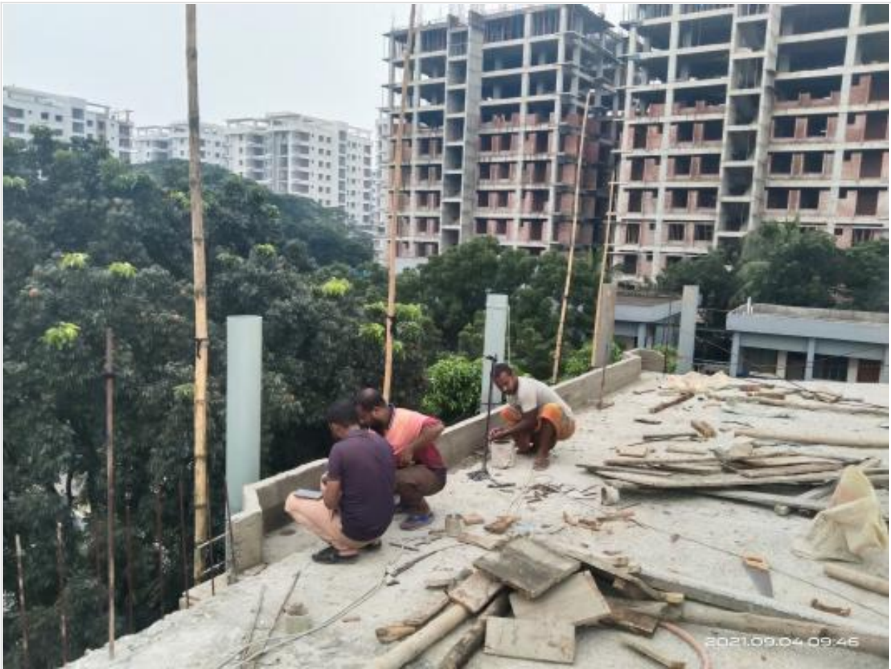
Roof top Gutter work on 04-09-21
