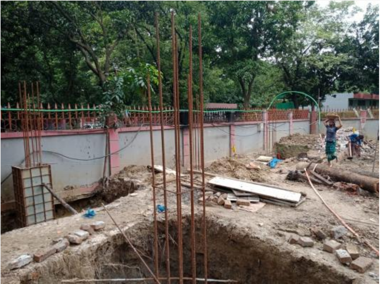
Substation-Generator Room-Excavation on 27-06-21
