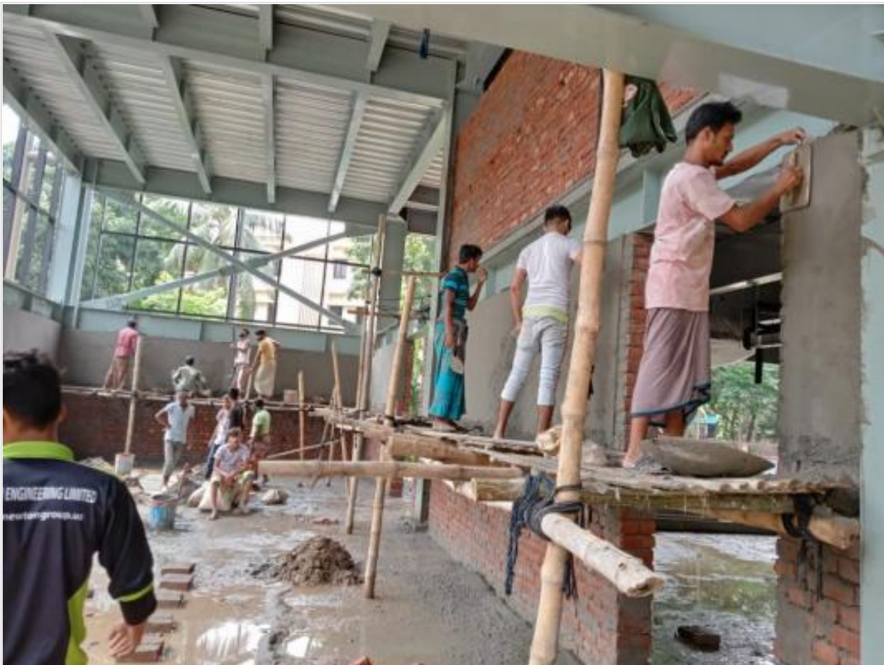
GF Mezzanine Shear Wall Plasteing on 09-08-21
