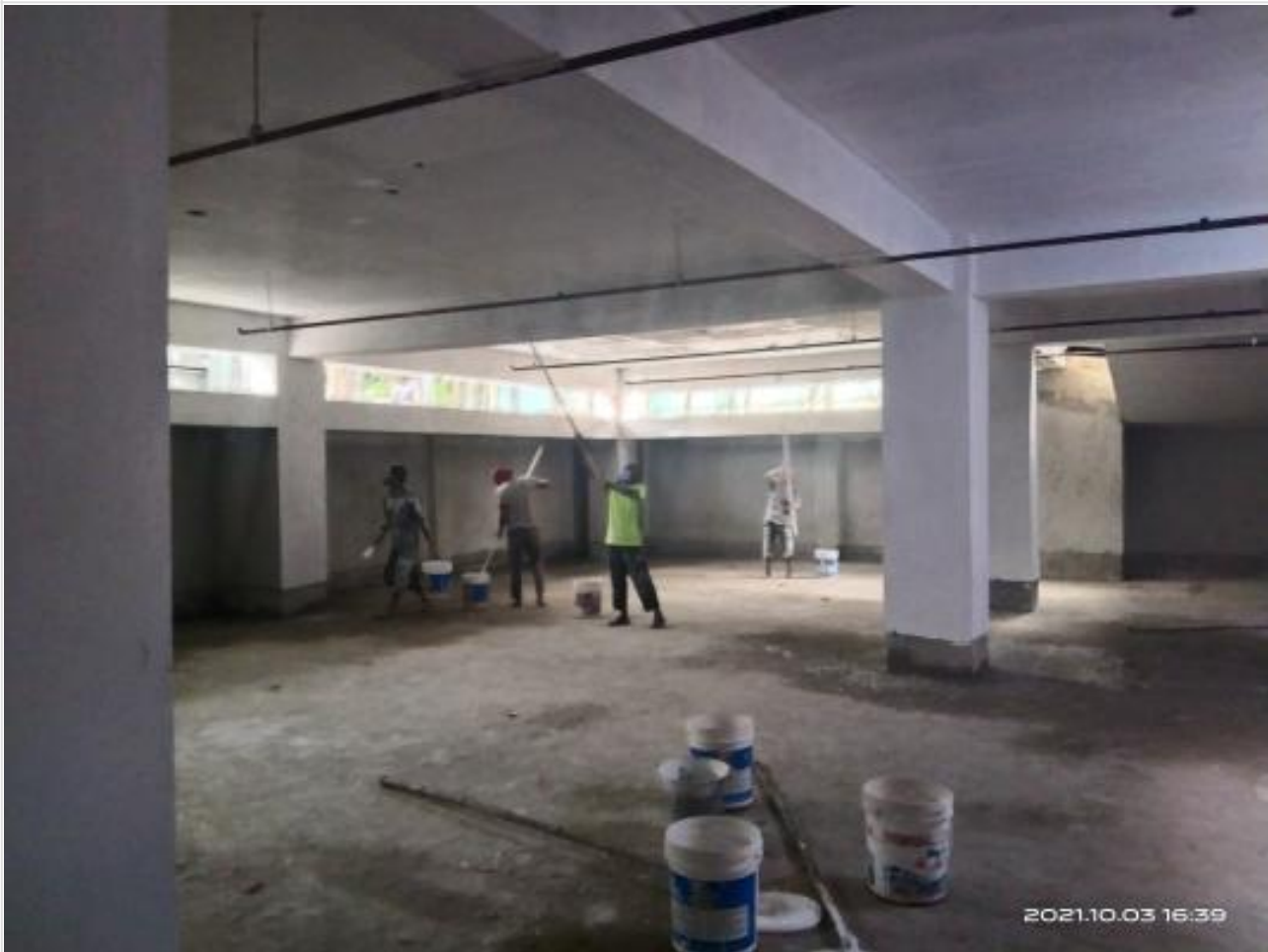
Basement wall and ceiling paint on 03-10-21
