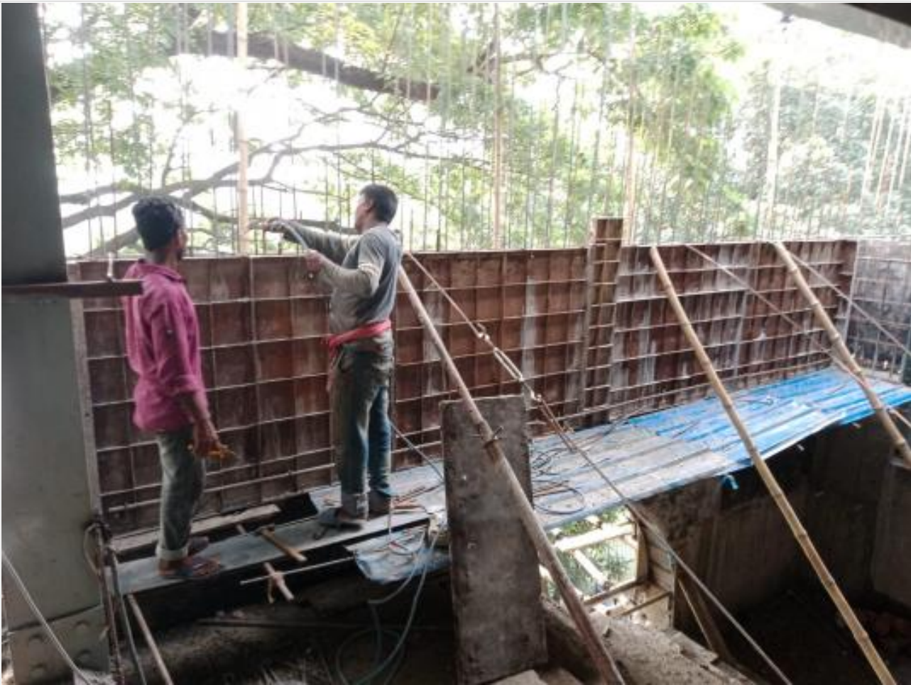
Stair RCC wall shuttering and casting on 12-10-21
