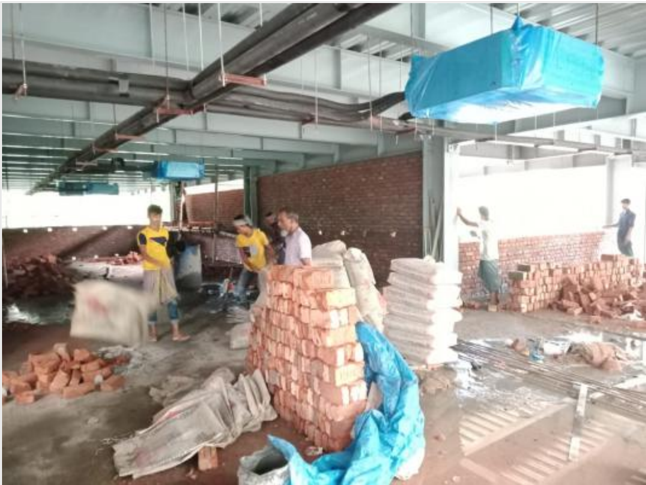
GF merzzanine brick work on 03-08-21
