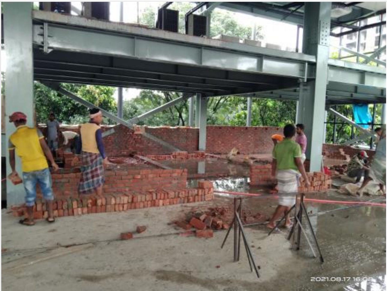
GF brick work on 17-08-21
