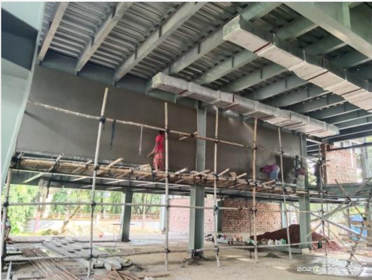
GF Mezzanine plaster work on 07-08-21
