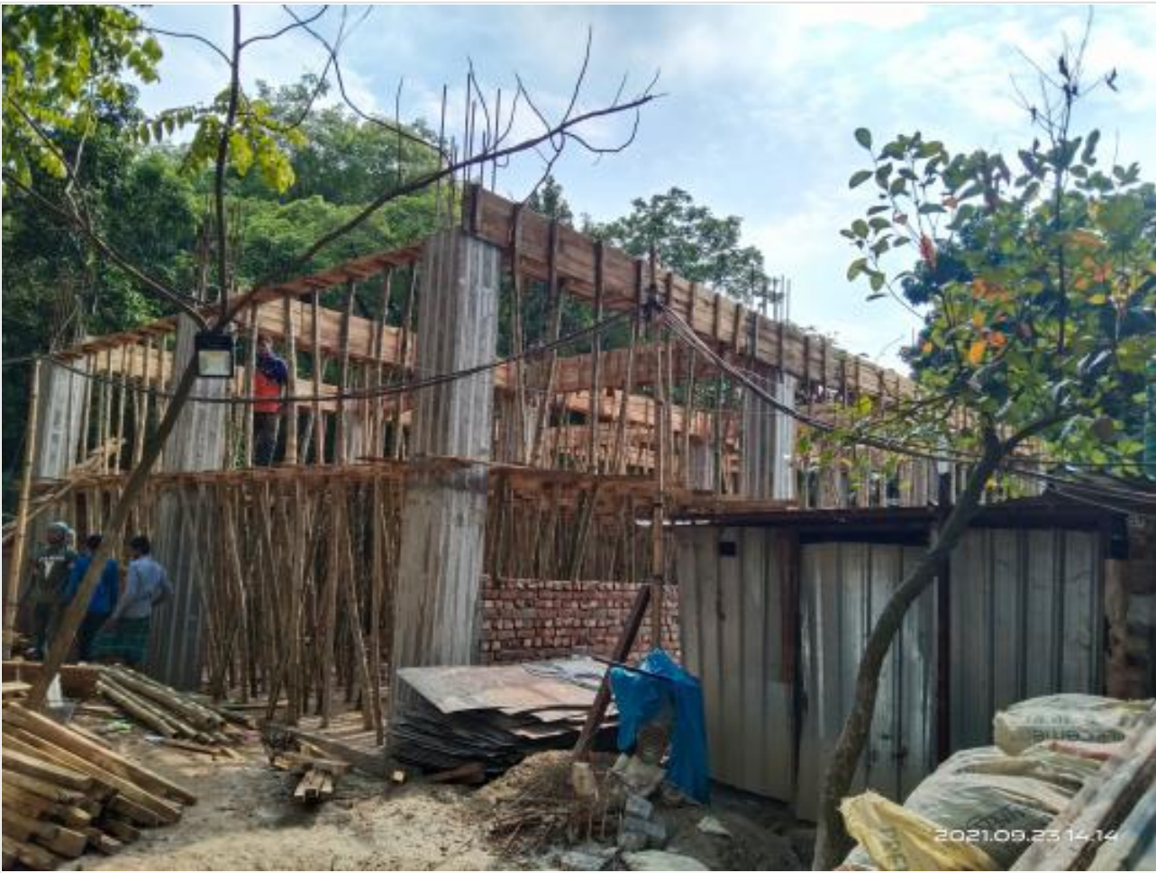
Generator room shuttering work on 23-09-21
