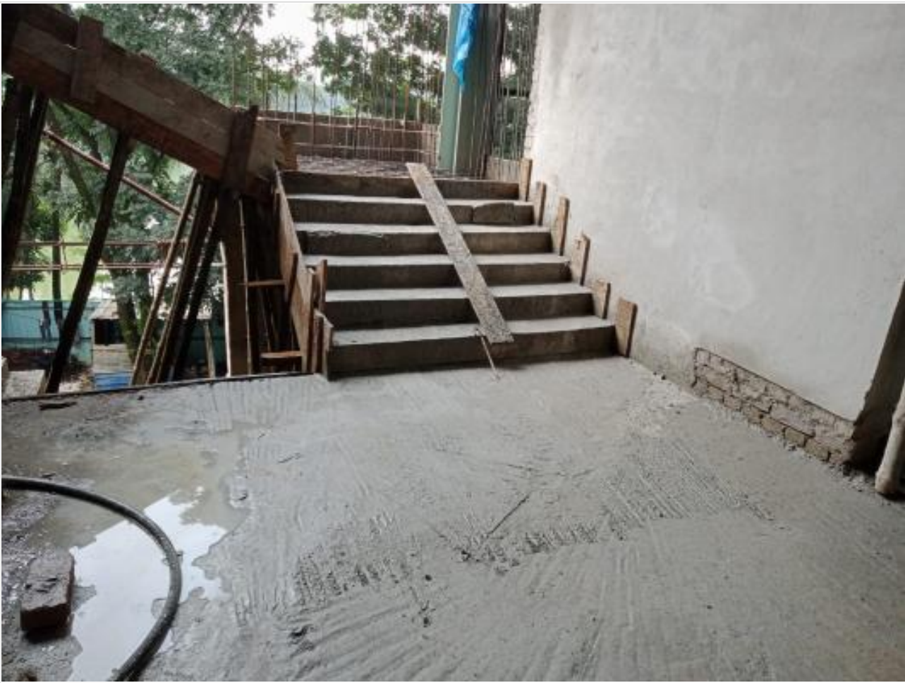
Stair casting on 05-10-21
