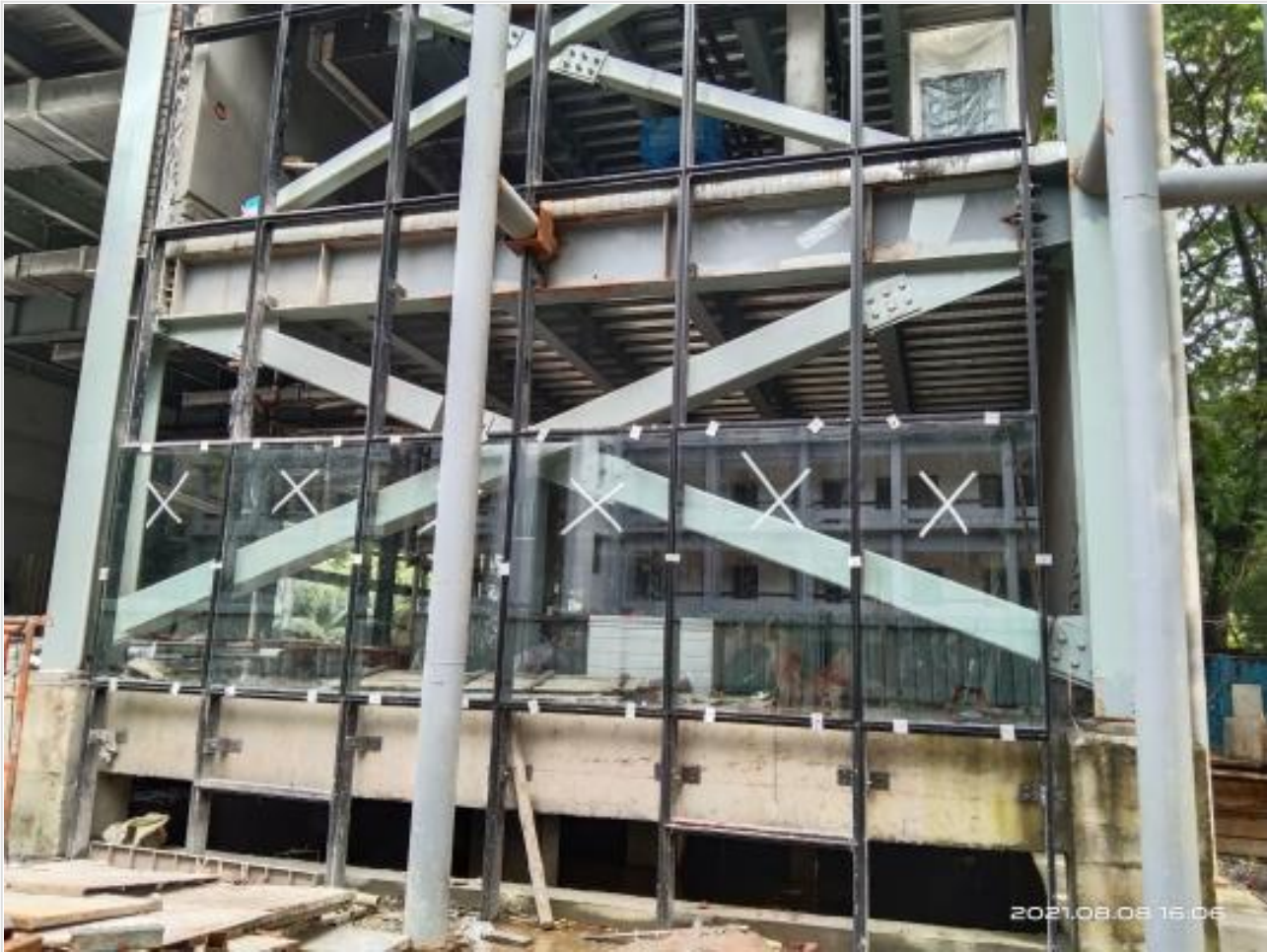
GF Glass fixing (31 sqm)=334 sft on 08-08-21
