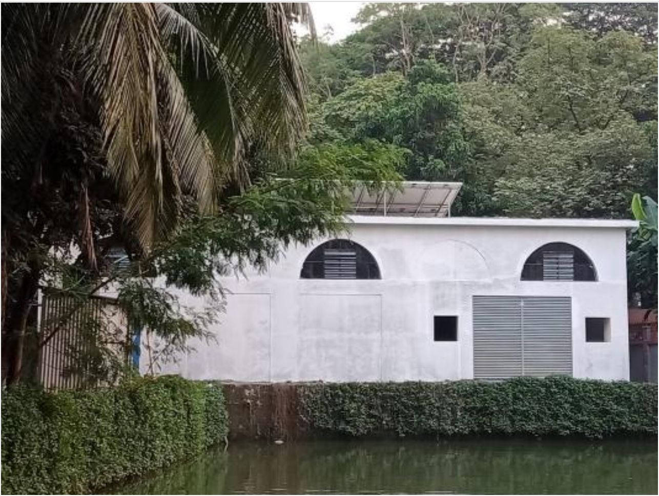
Generator room on 13-12-21
