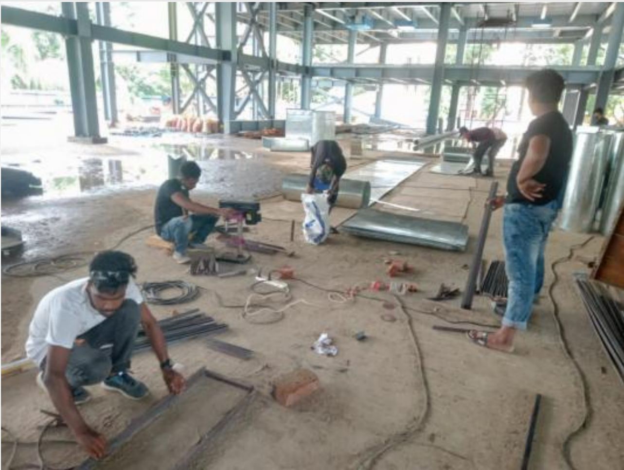
AC Duct Making on 19-05-21
