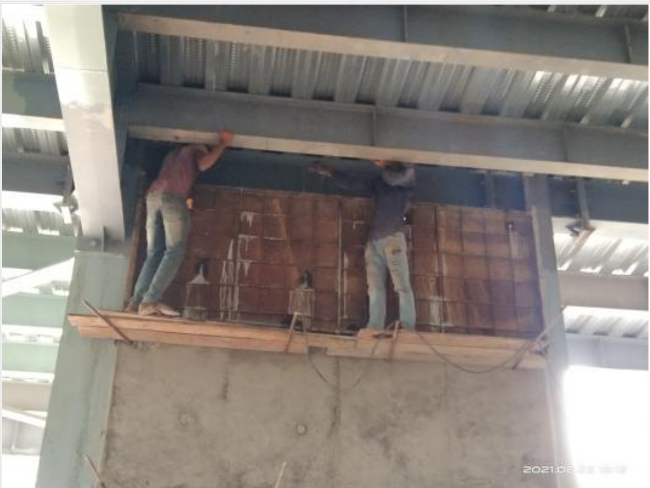
GF Stair Shuttering on 23-08-21
