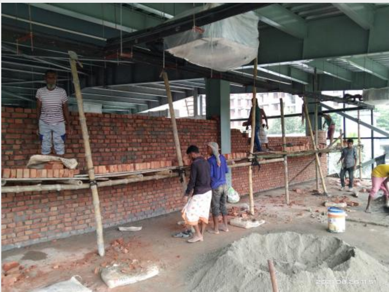
FFM brick work on 26-08-21
