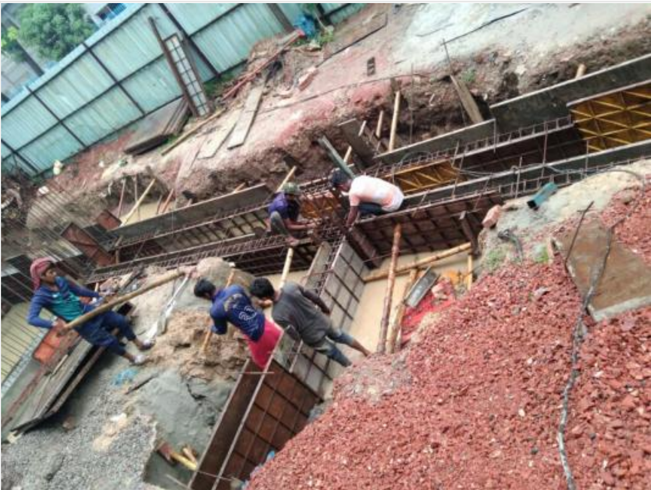
Porch Grade Beam Shuttering on 09-06-21
