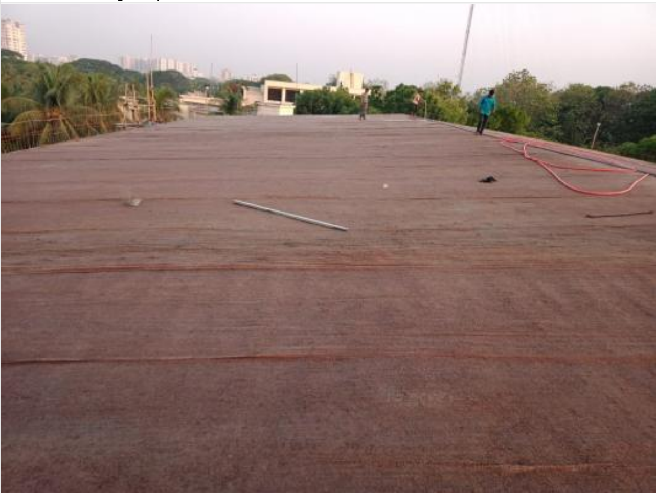
Hessain Cloth Covering after Concreting on 07-05-21
