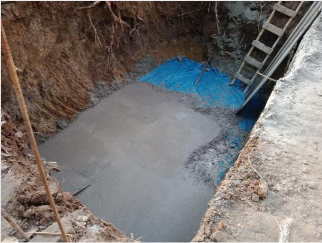
Septic tank cc work on 15-09-21
