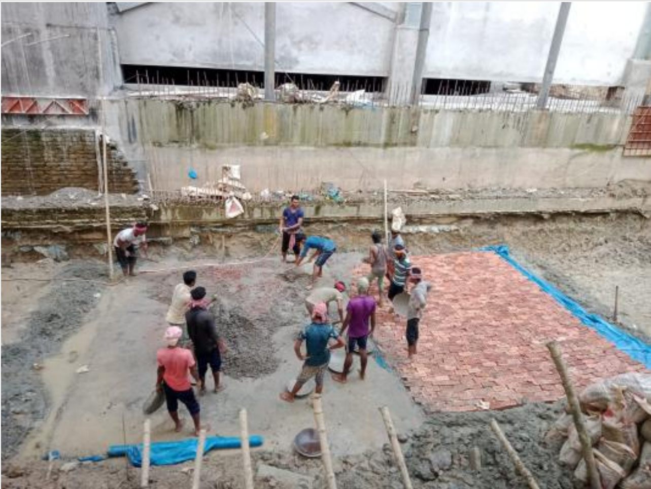
Fire tank base cc casting on 11-09-21
