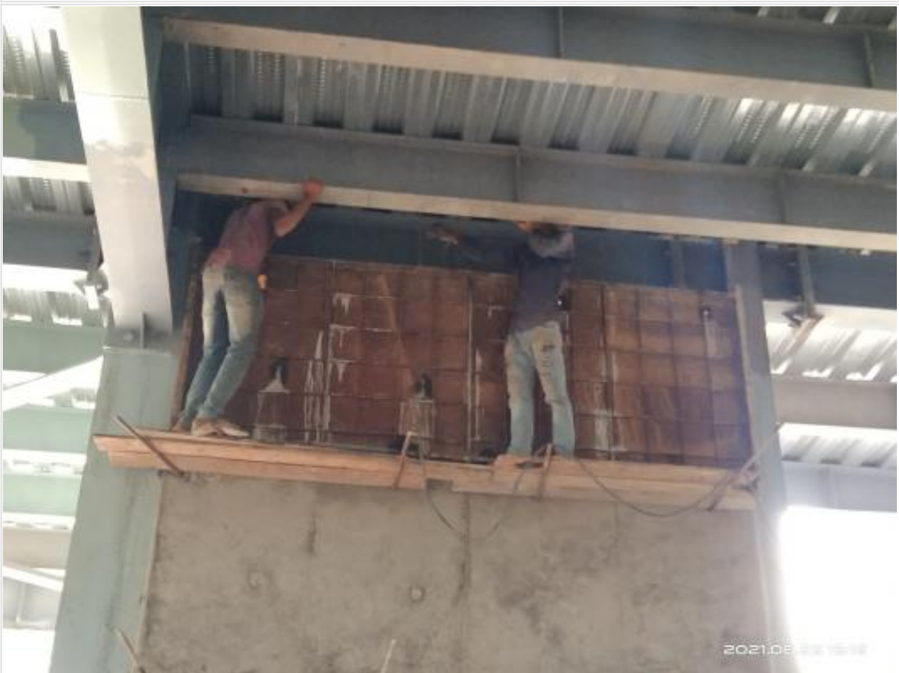
GF Stair Shuttering on 23-08-21
