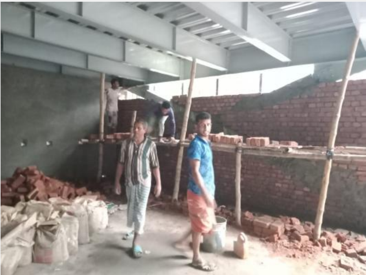
GF brick work on 10-08-21
