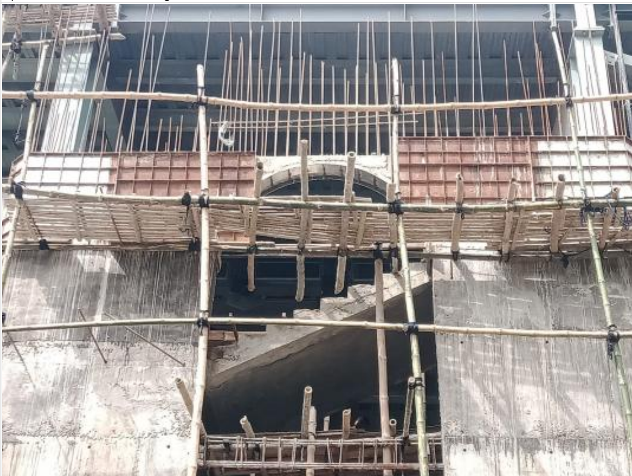
Stair Arch Casting (stair no. 2) on 17-09-21
