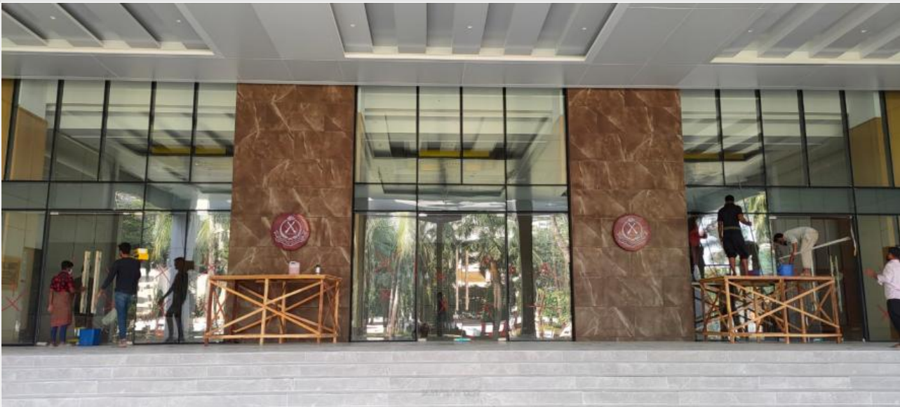
Main Entrance on 17-12-21
