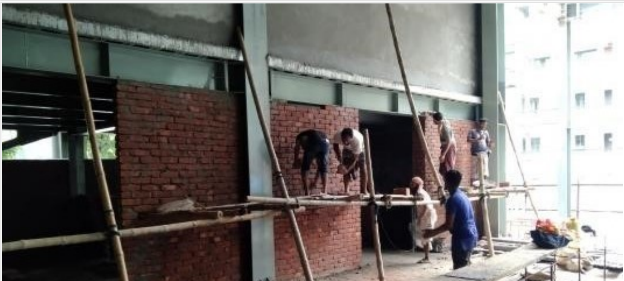
GF Brick work on 14-08-21
