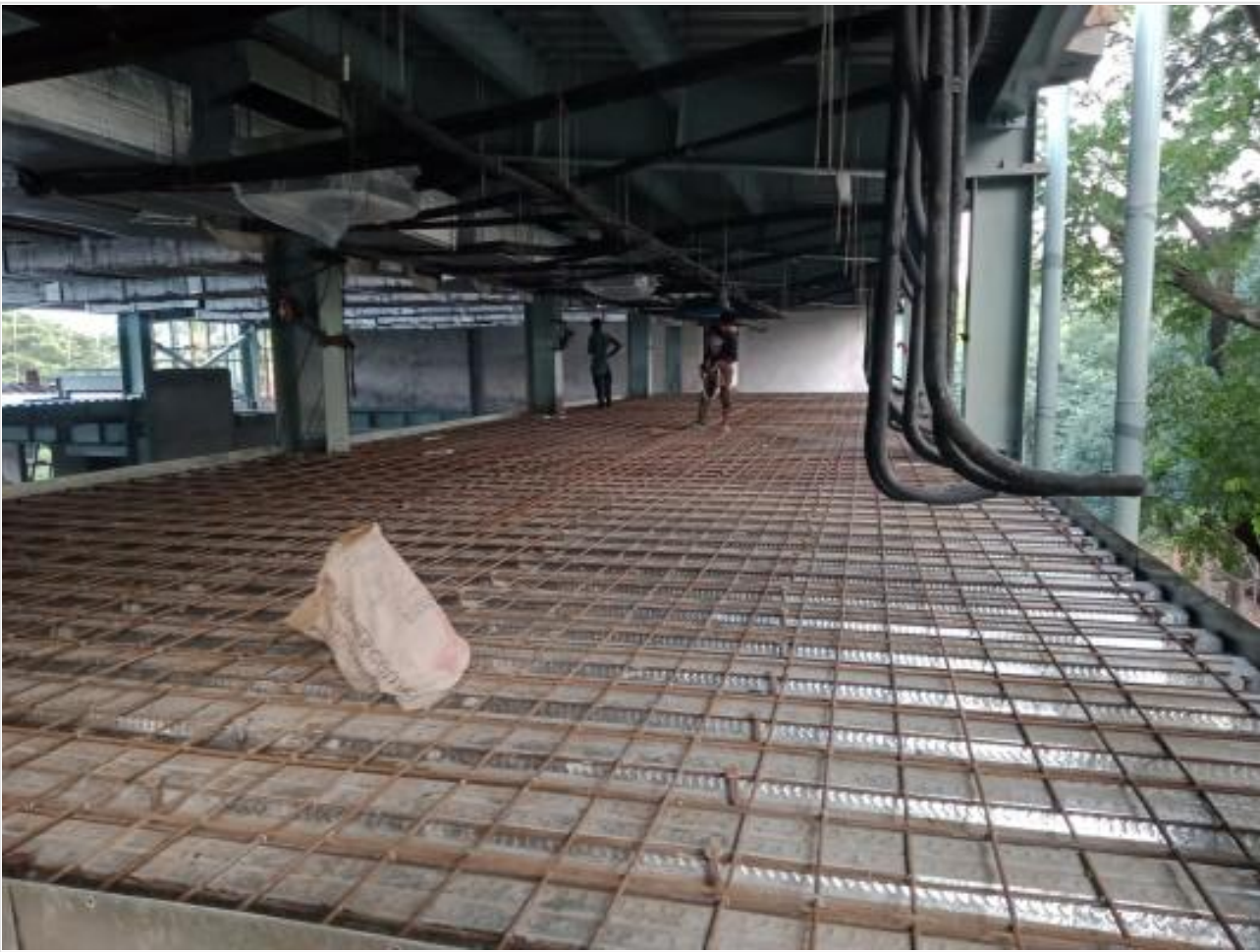
Rod binding at 1st floor mezzanine on 26-09-21
