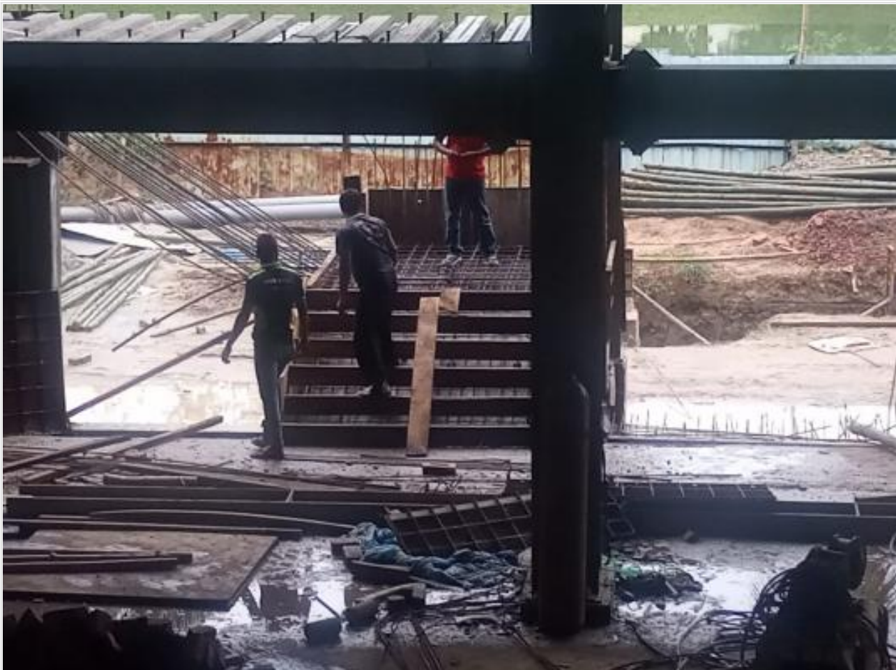
Ground Floor Stair Re-bar work on 01-07-21
