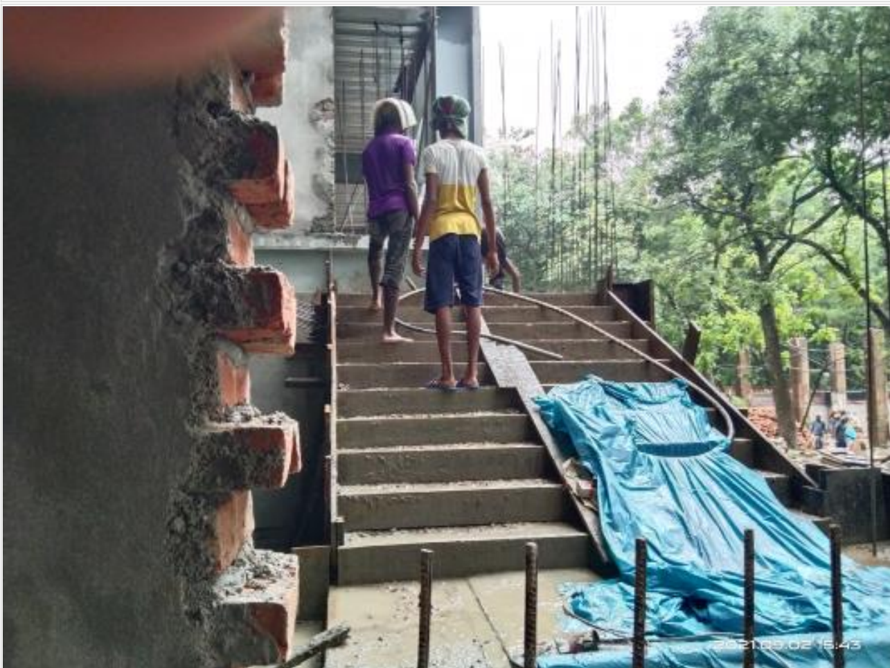
Grond floor stair casting on 02-09-21
