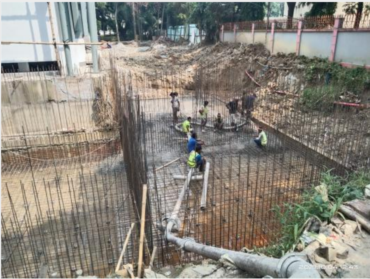
Fire tank base casting on 04-10-21
