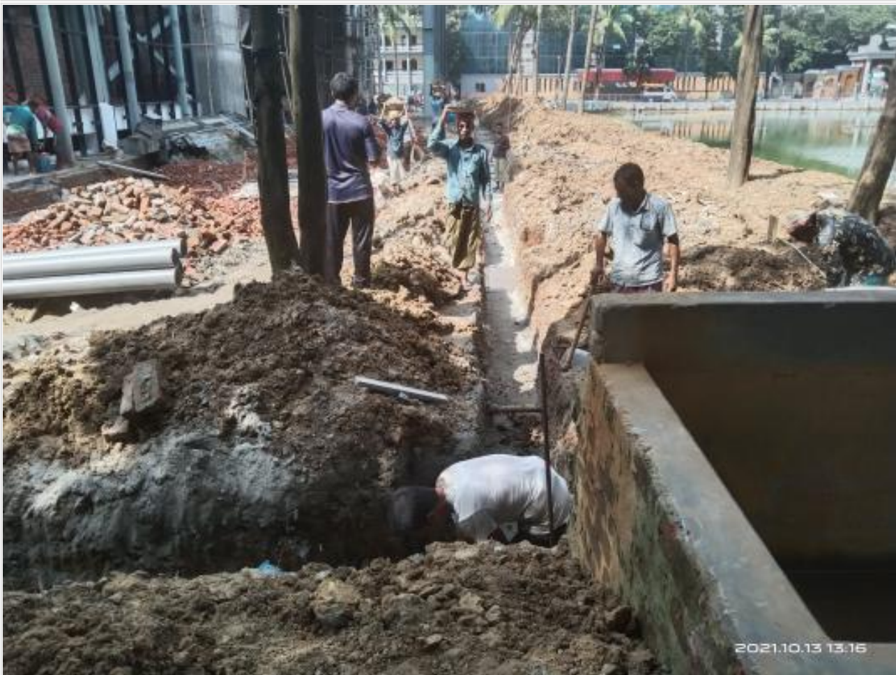
Outside drain work with pit on 13-10-21
