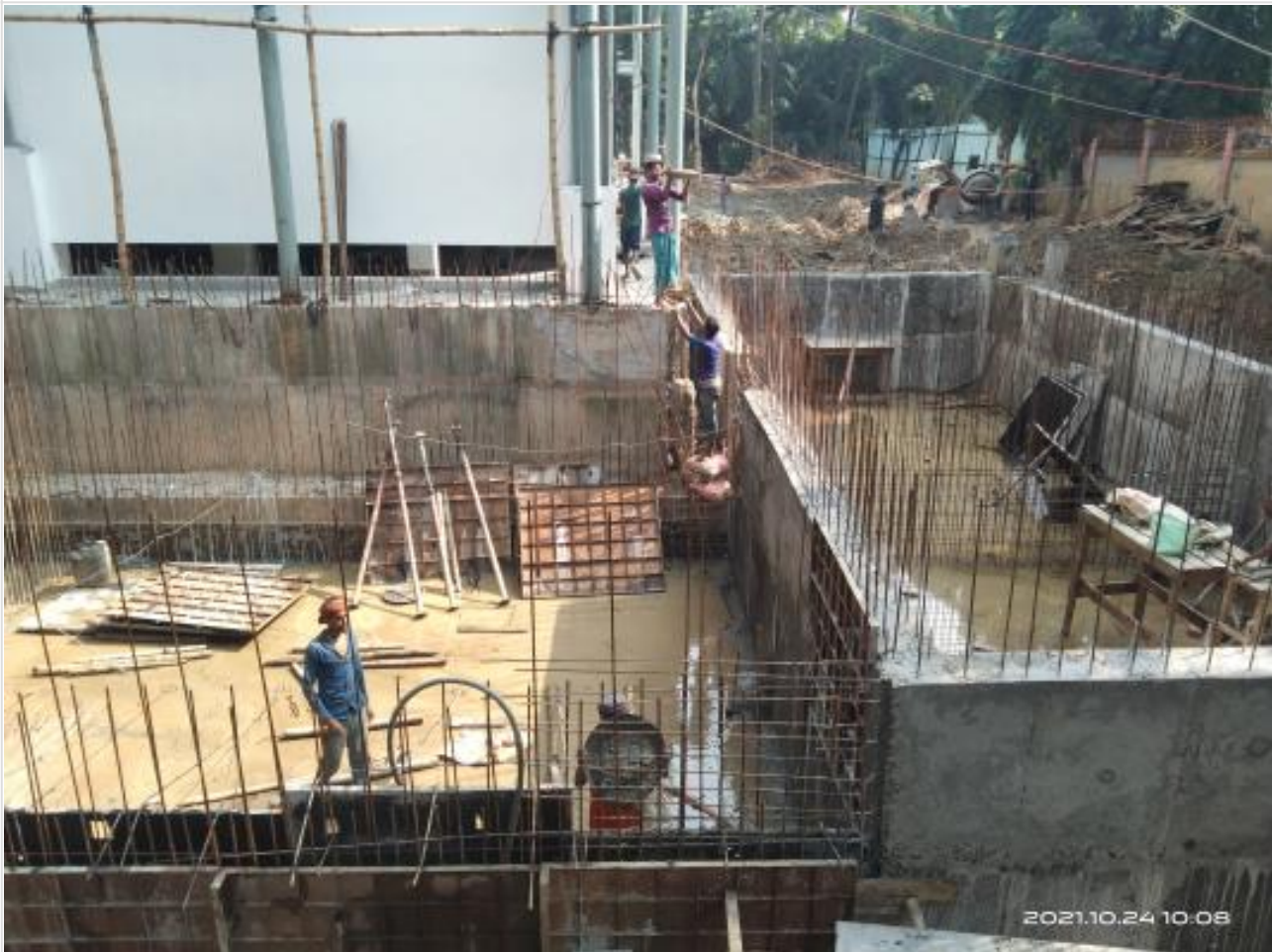
Fire tank wall casting on 24-10-21
