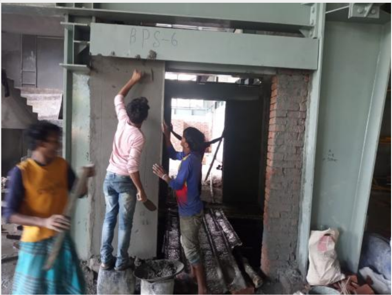
Lift door wall plaster on 22-09-21
