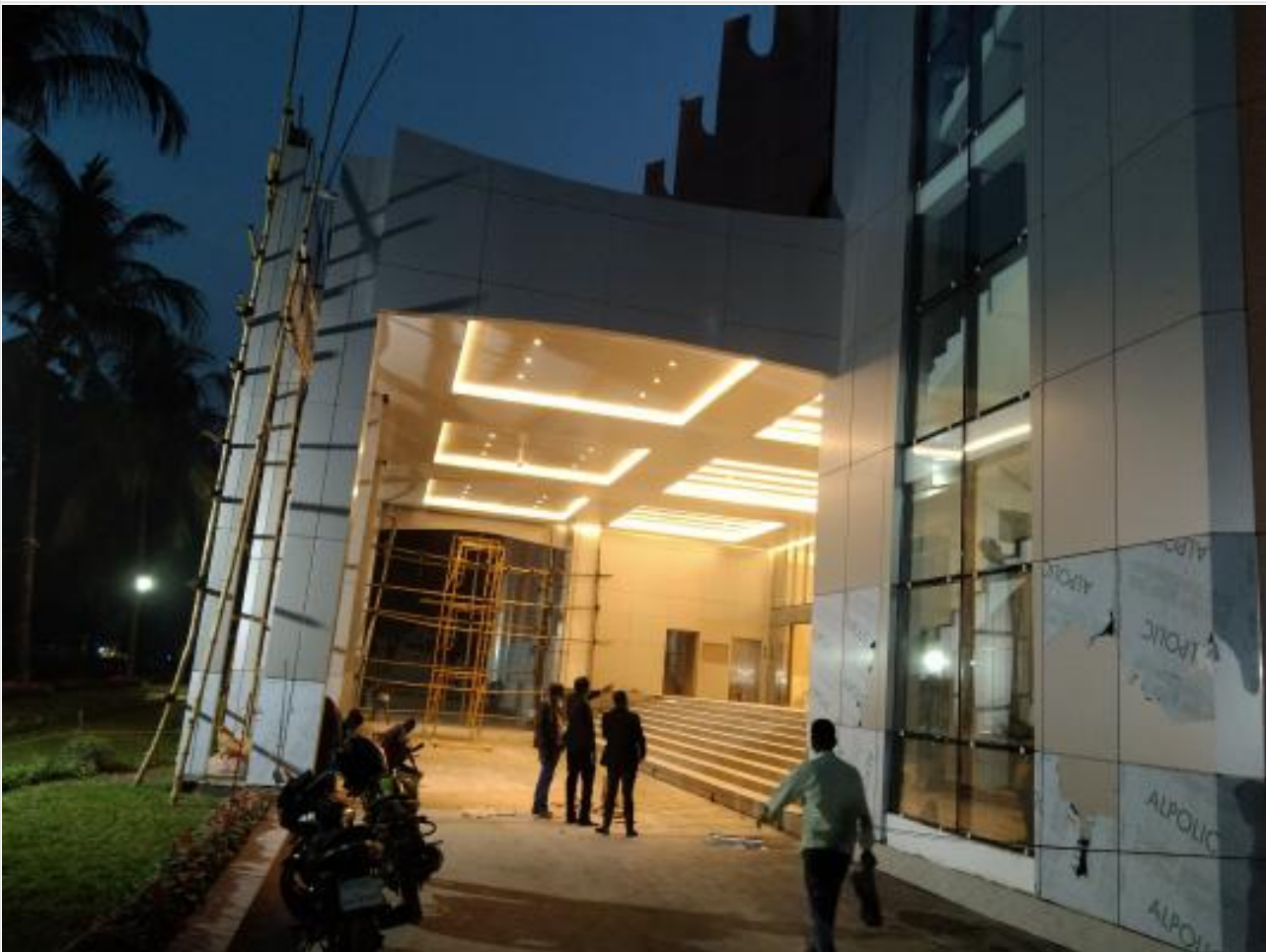
Interior work on 15-12-21
