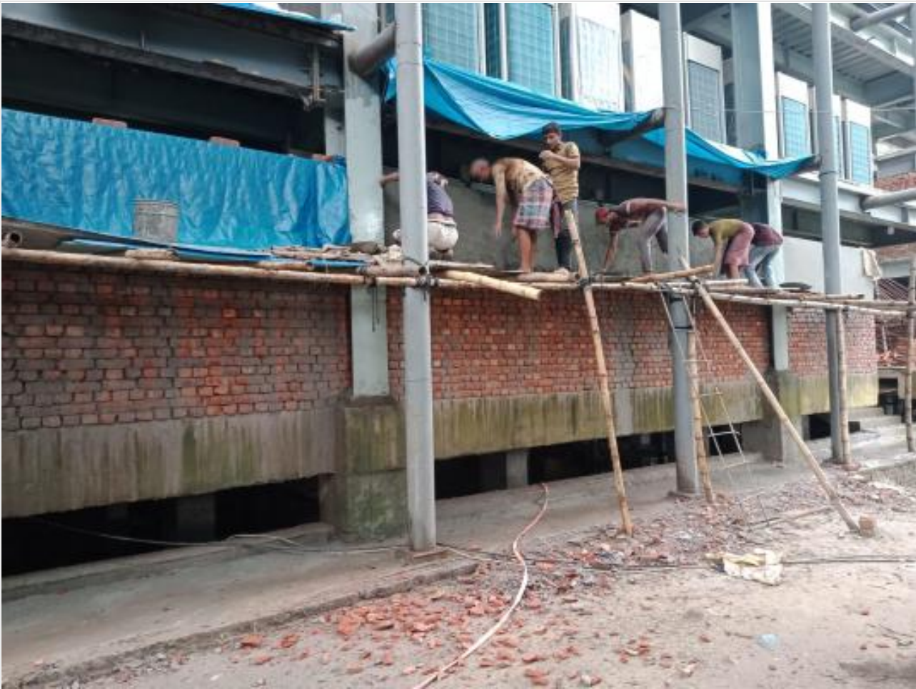
GF Brick wall on 11-08-21
