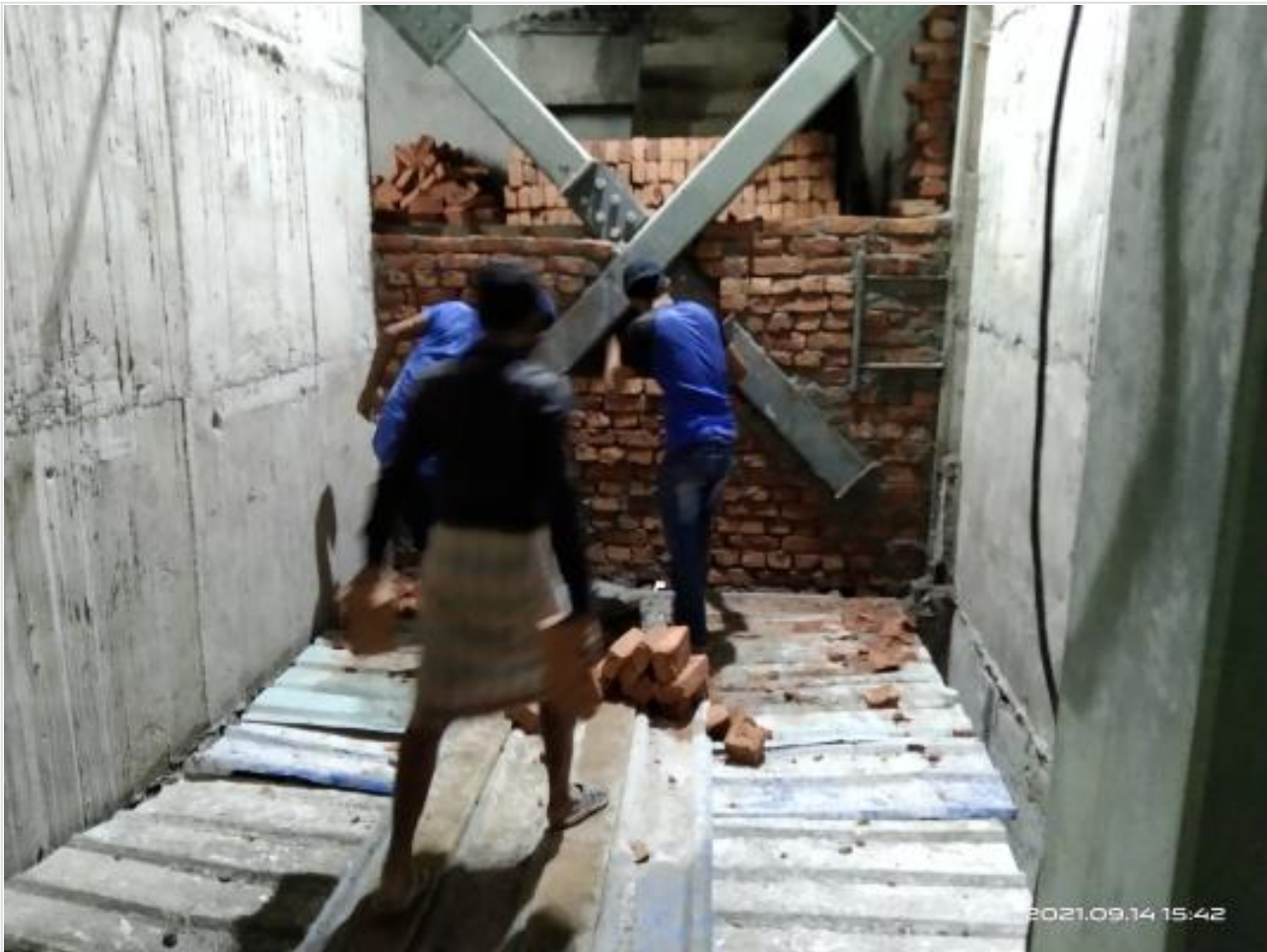
Brick work for lift on 14-09-21
