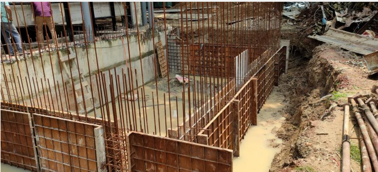
Domestic Water Tank Wall Shuttering on 02-06-21
