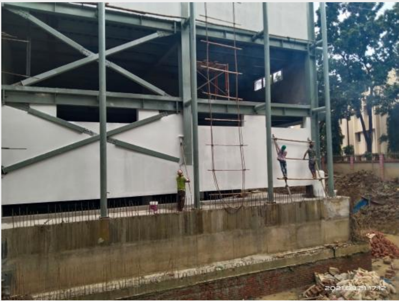
Exterior wall painting work on 21-09-21
