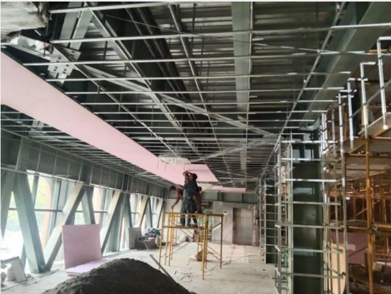
First floor ceiling work on 05-01-22
