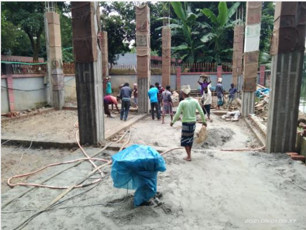
Sub-Station room floor Development work on 01-09-21
