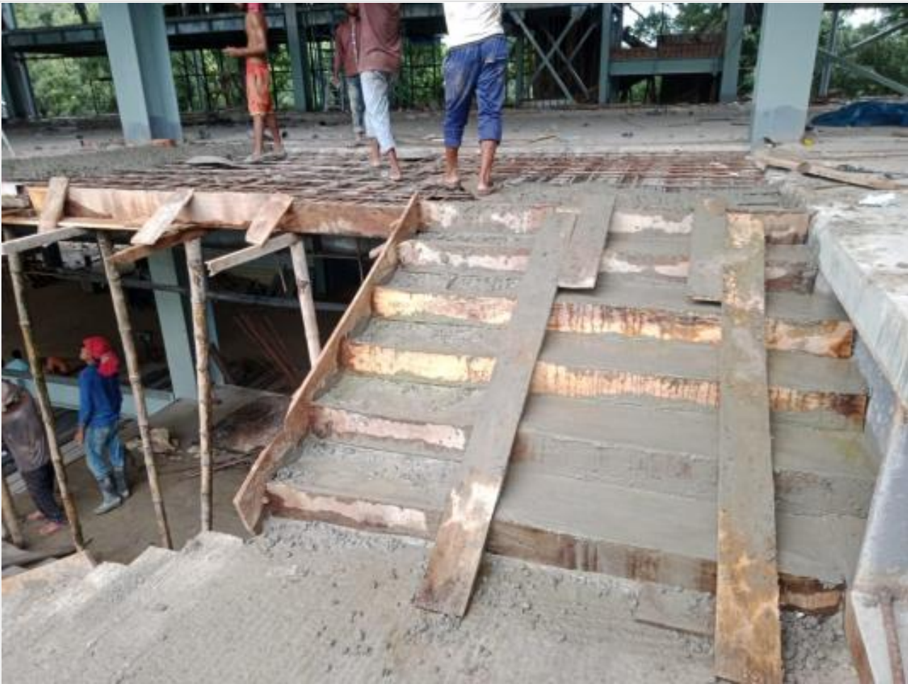
Gr.Floor Mezzanine Stair Concreting on 18-07-21
