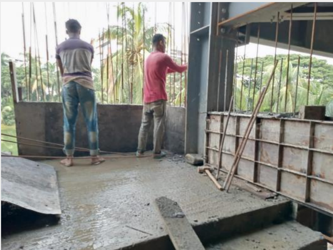
1st floor stair rod binding on 01-08-21
