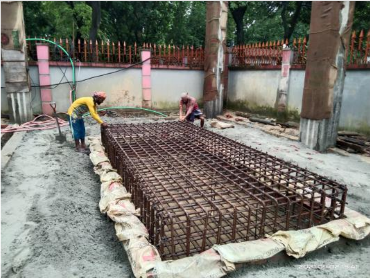
Generator foundation rod binding on 02-09-21
