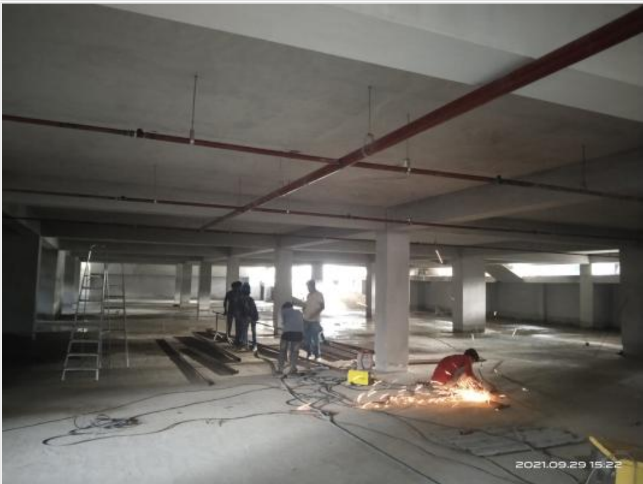
Fire pipe fitting at basement floor on 29-09-21
