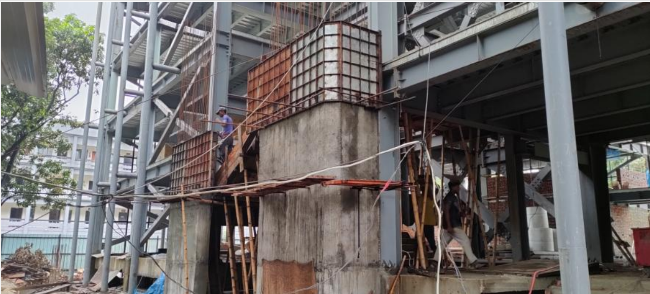
GF Mezzanine Stair Wall Concreting on 16-06-21
