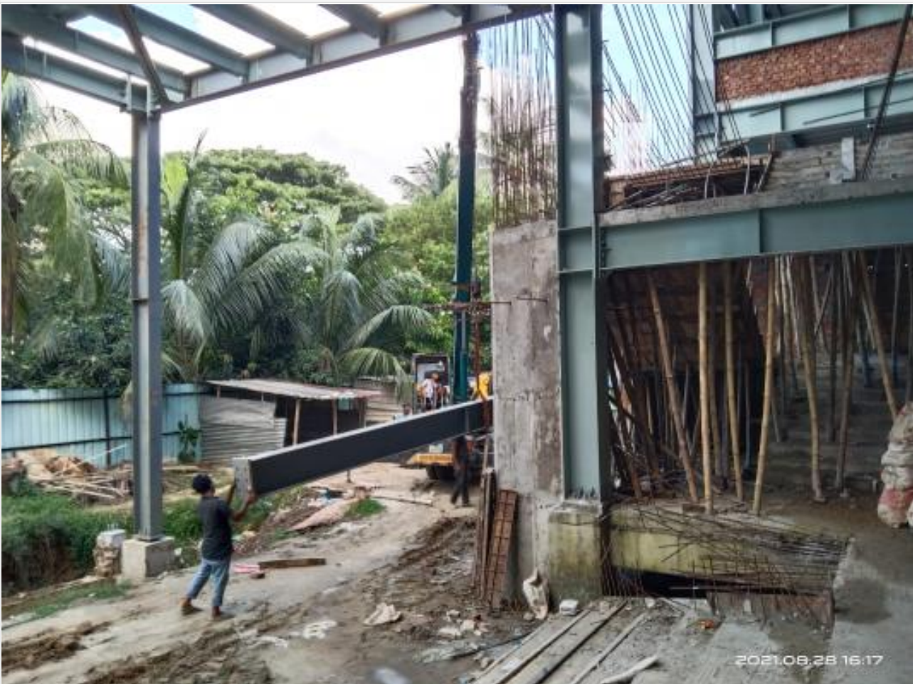
Steel beam shifting on 28-08-21
