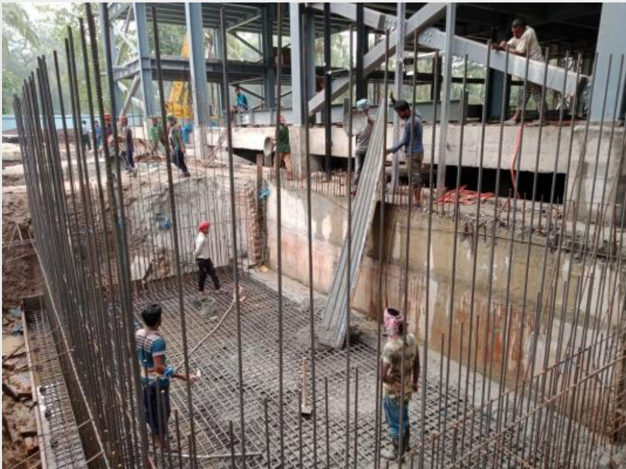
Domestic Water Tank Base concreting on 03-05-21
