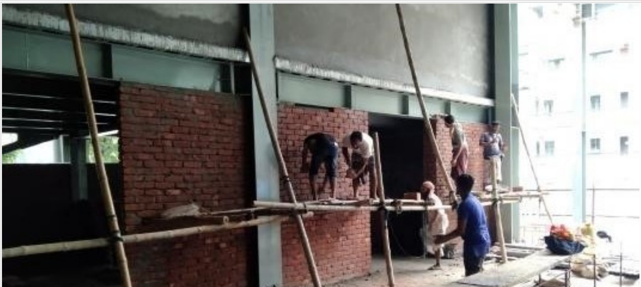
GF Brick work on 14-08-21
