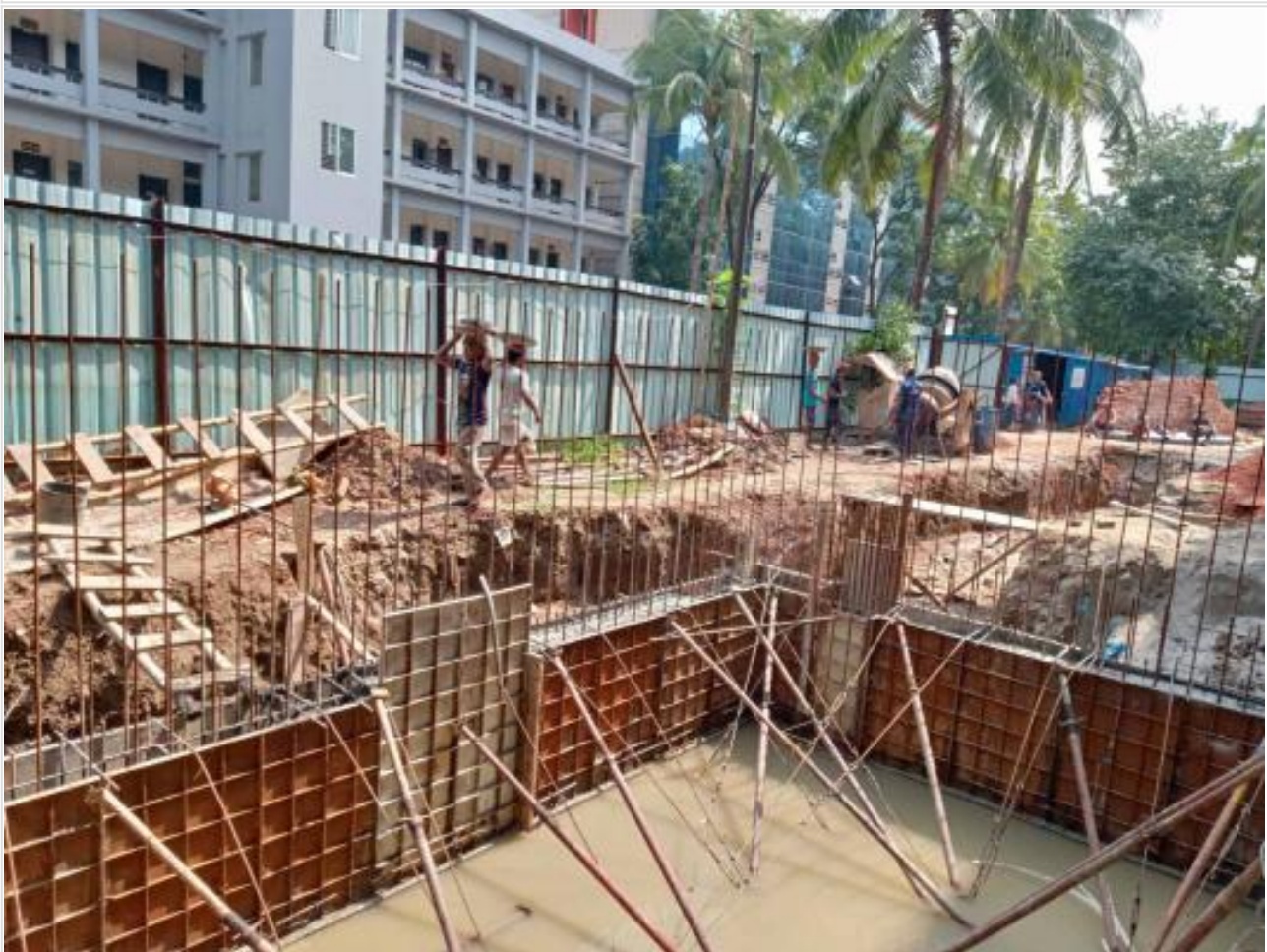
Domestic Water Tank-1st Lift Concreting on 04-06-21
