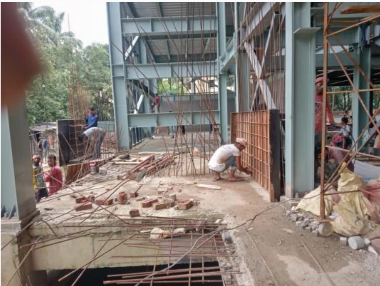
GF Stair work (stair no. 3) on 11-08-21
