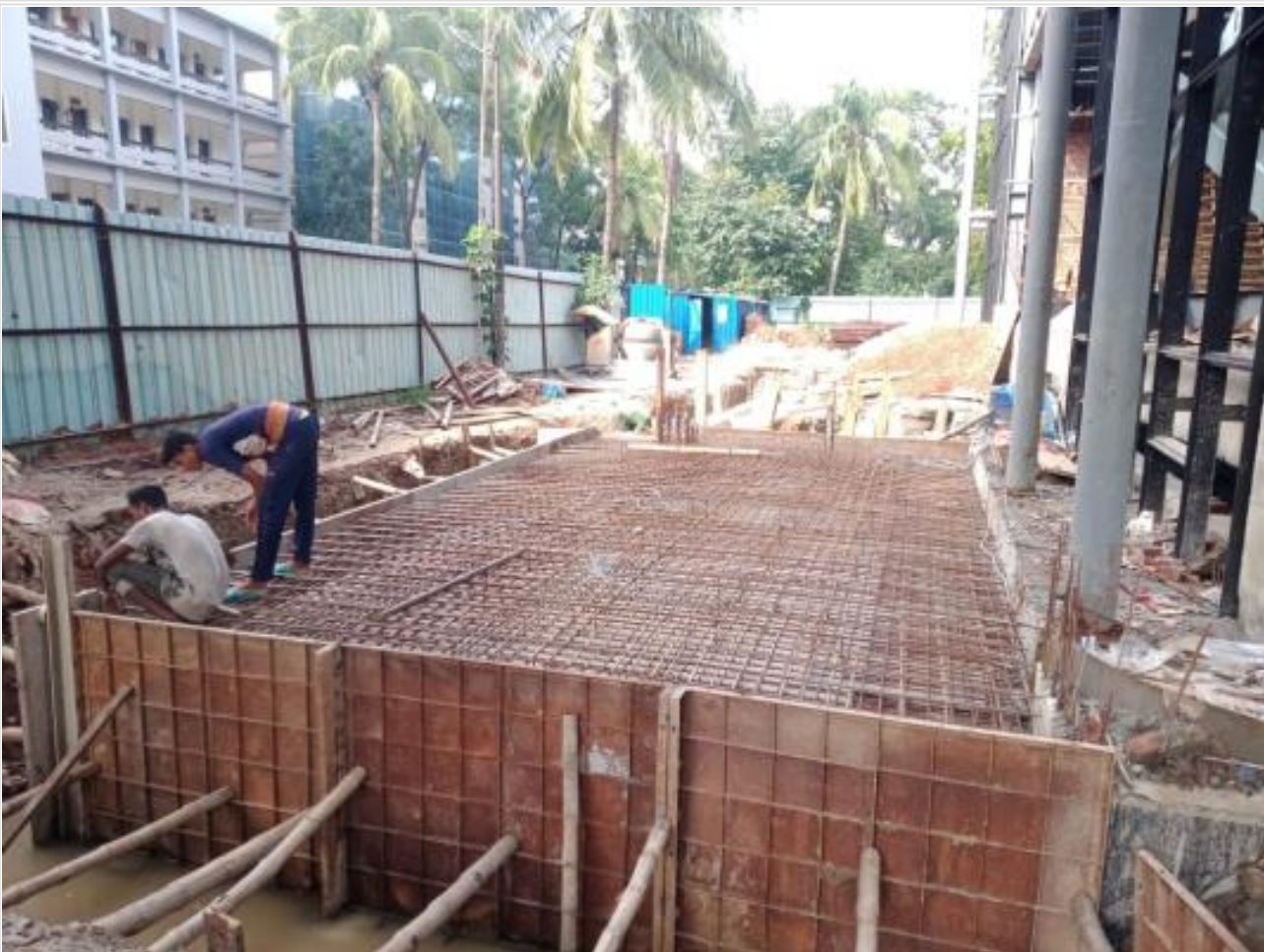
Domestic Water Tank Slab Re-barwork on 23-06-21
