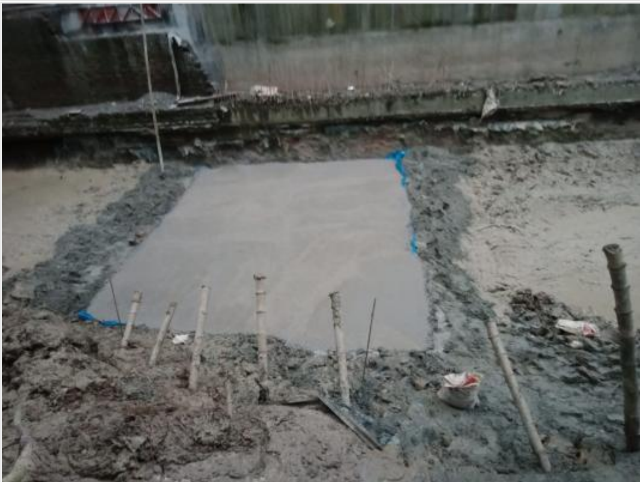
Fire Tank CC Base Casting on 10-09-21
