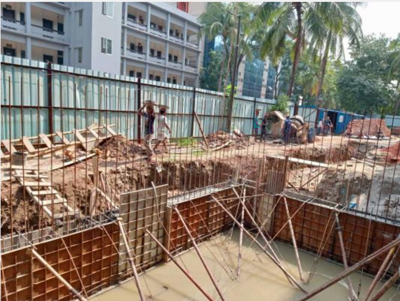
Domestic Water Tank-1st Lift Concreting on 04-06-21
