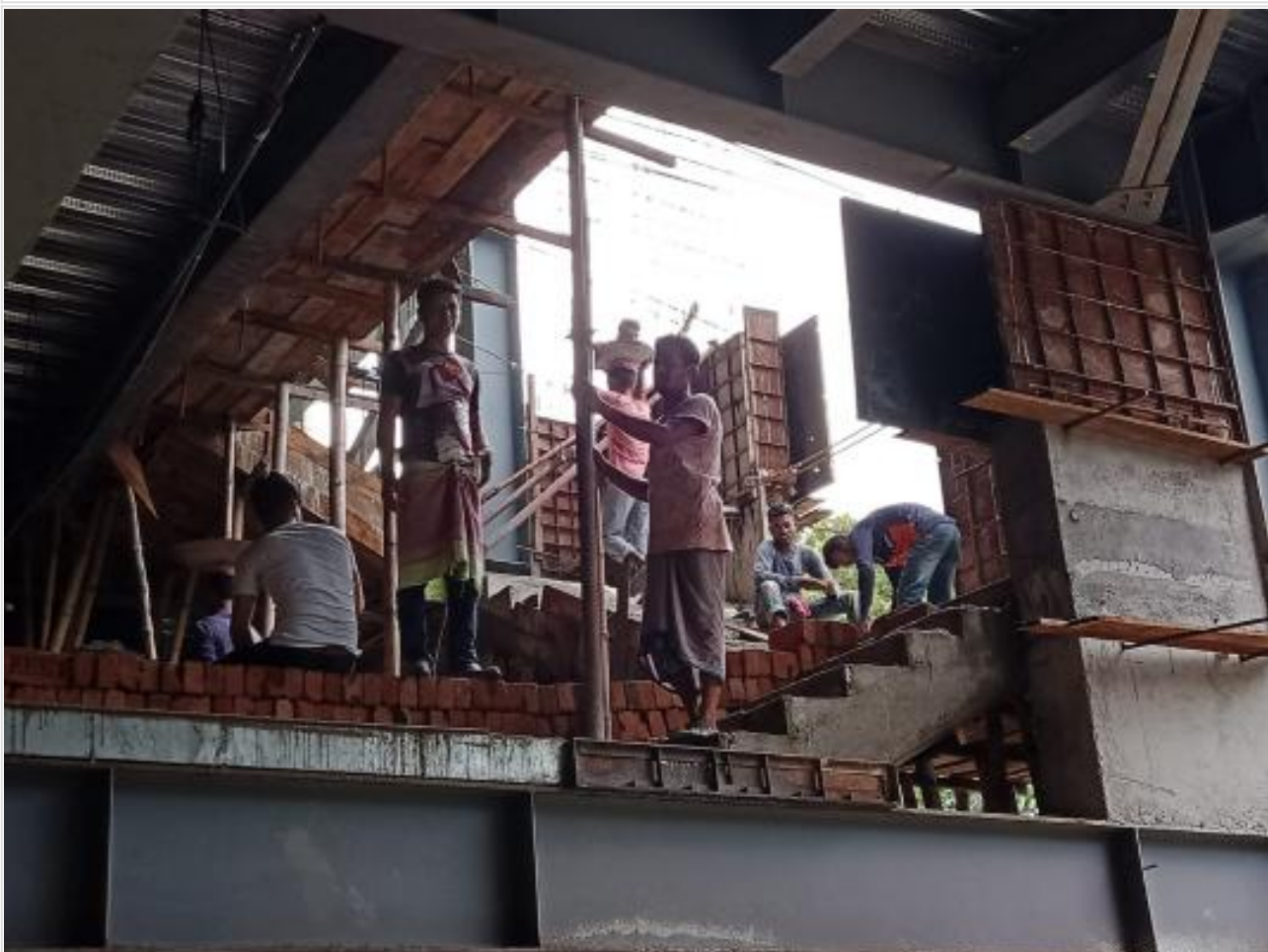
GF Mazzanine stair wall casting on 04-08-21
