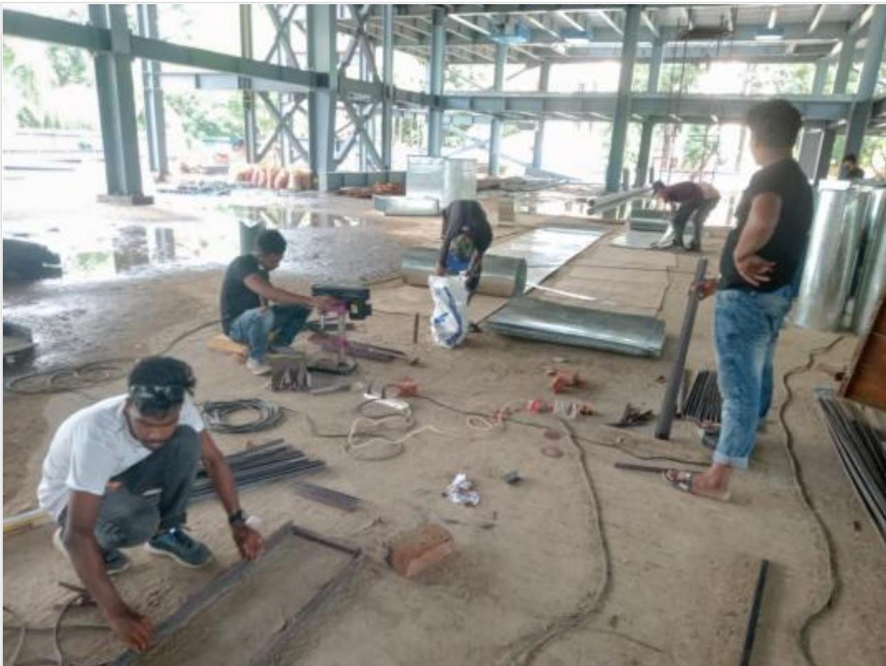
AC Duct Making on 19-05-21
