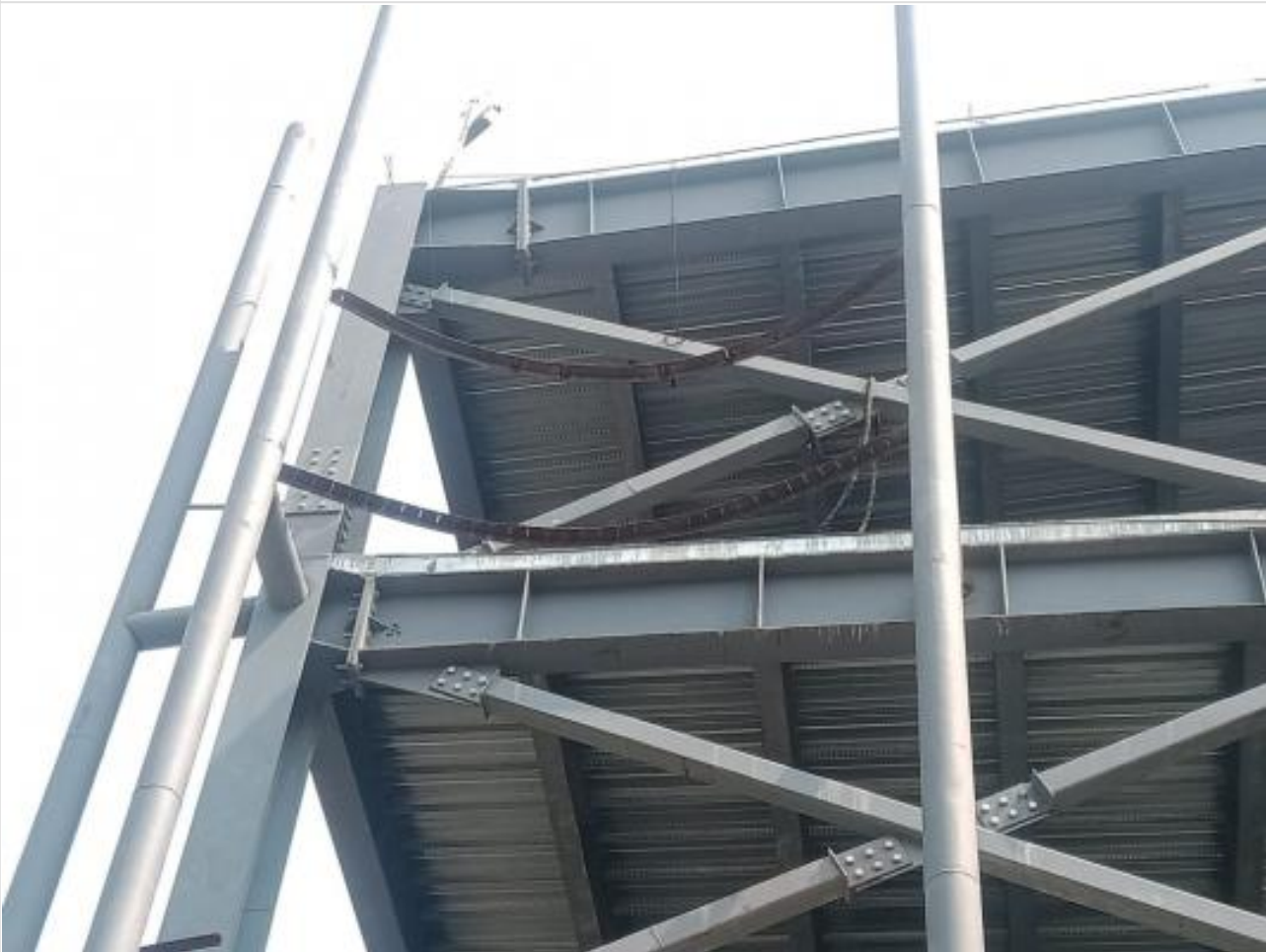
ACP Post Setting on 05-05-21
