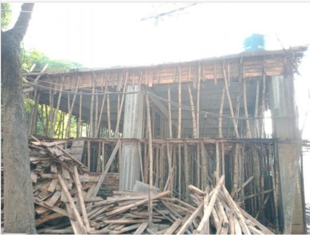
Generator room shutter remove on 16-10-21
