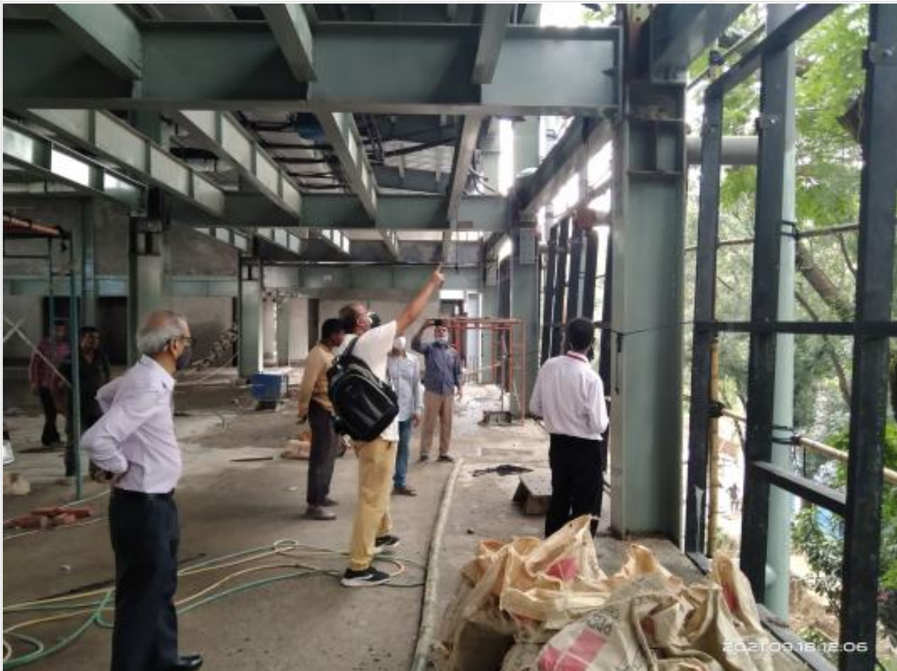
Consultent site visit (Architectural and on 18-09-21
