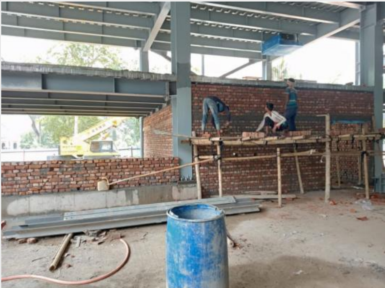
Ground Floor Brickwork on 11-05-21
