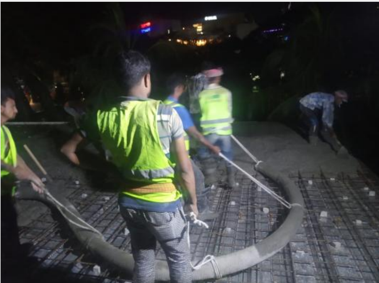
Canopy Casting on 08-09-21
