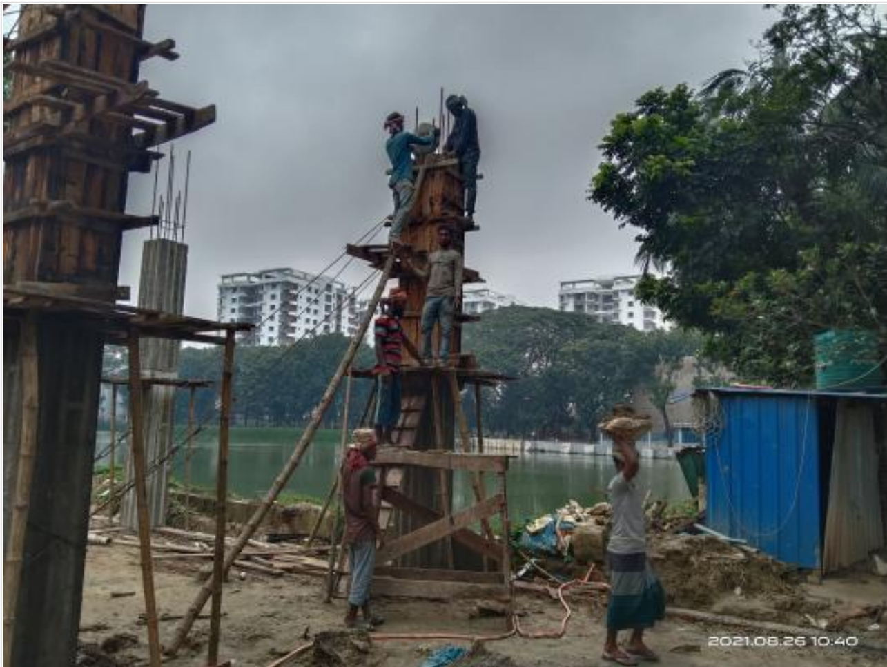
Generator room Column casting on 26-08-21
