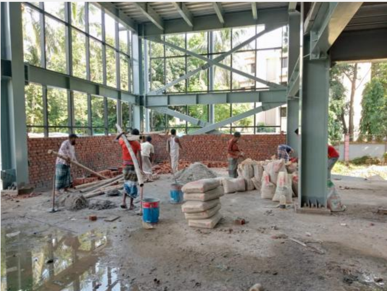
GF brick work on 05-08-21
