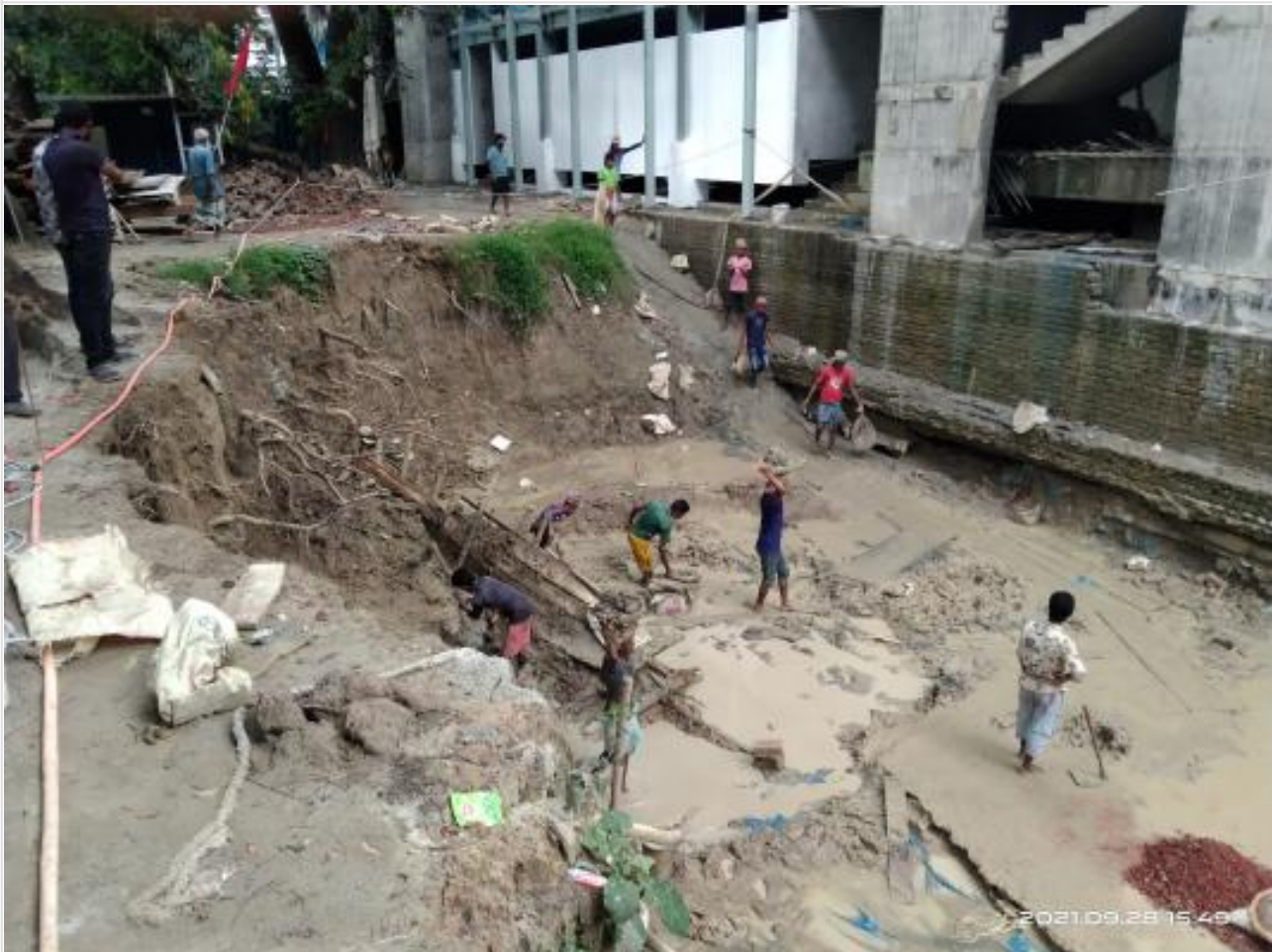
Fire tank base clay remove on 28-09-21
