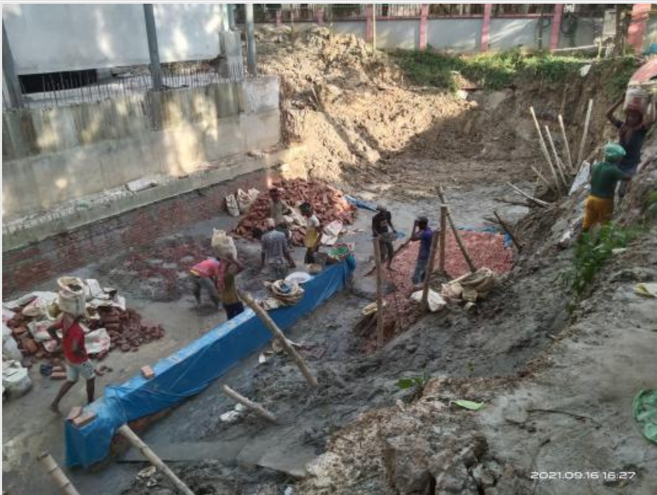
Fire tank cc work on 16-09-21
