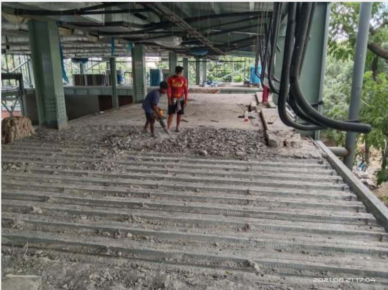
FF Mezzanine floor dismantling work on 21-08-21
