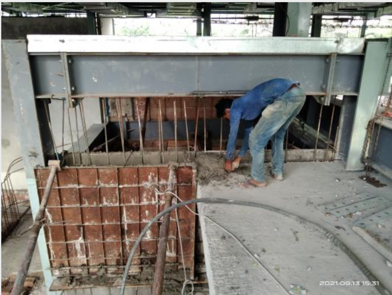
Lift wall casting on 13-09-21
