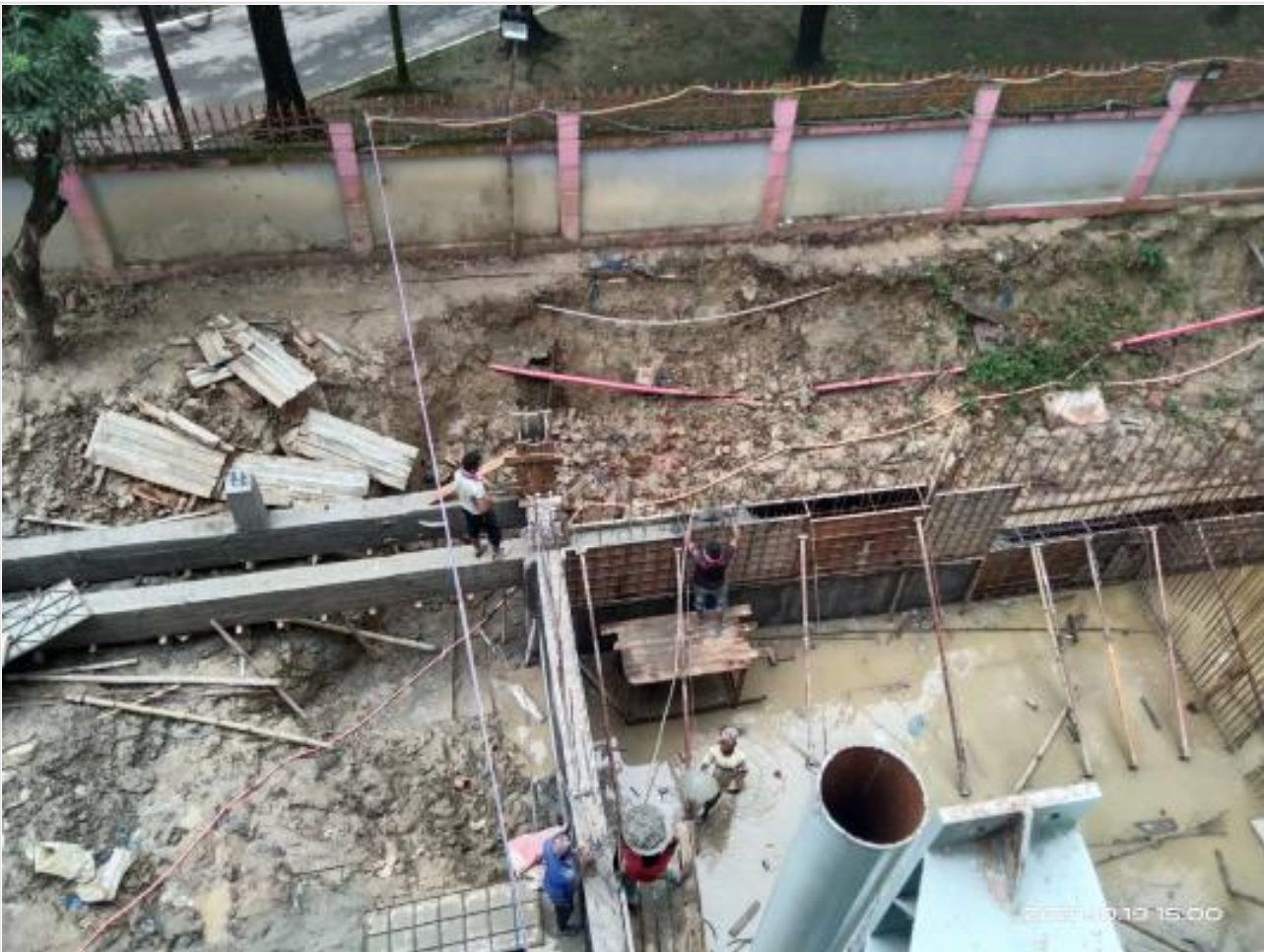
Fire Tank wall casting on 19-10-21
