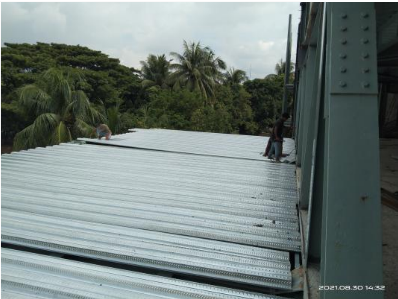
East Canopy decking sheet shitting on 30-08-21
