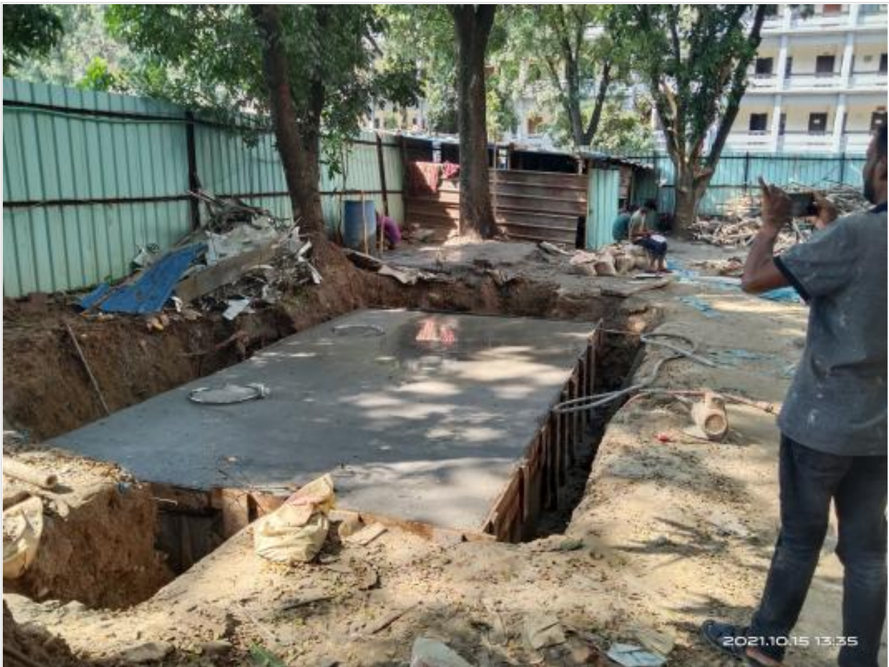
Septic tank top slab casting on 15-10-21
