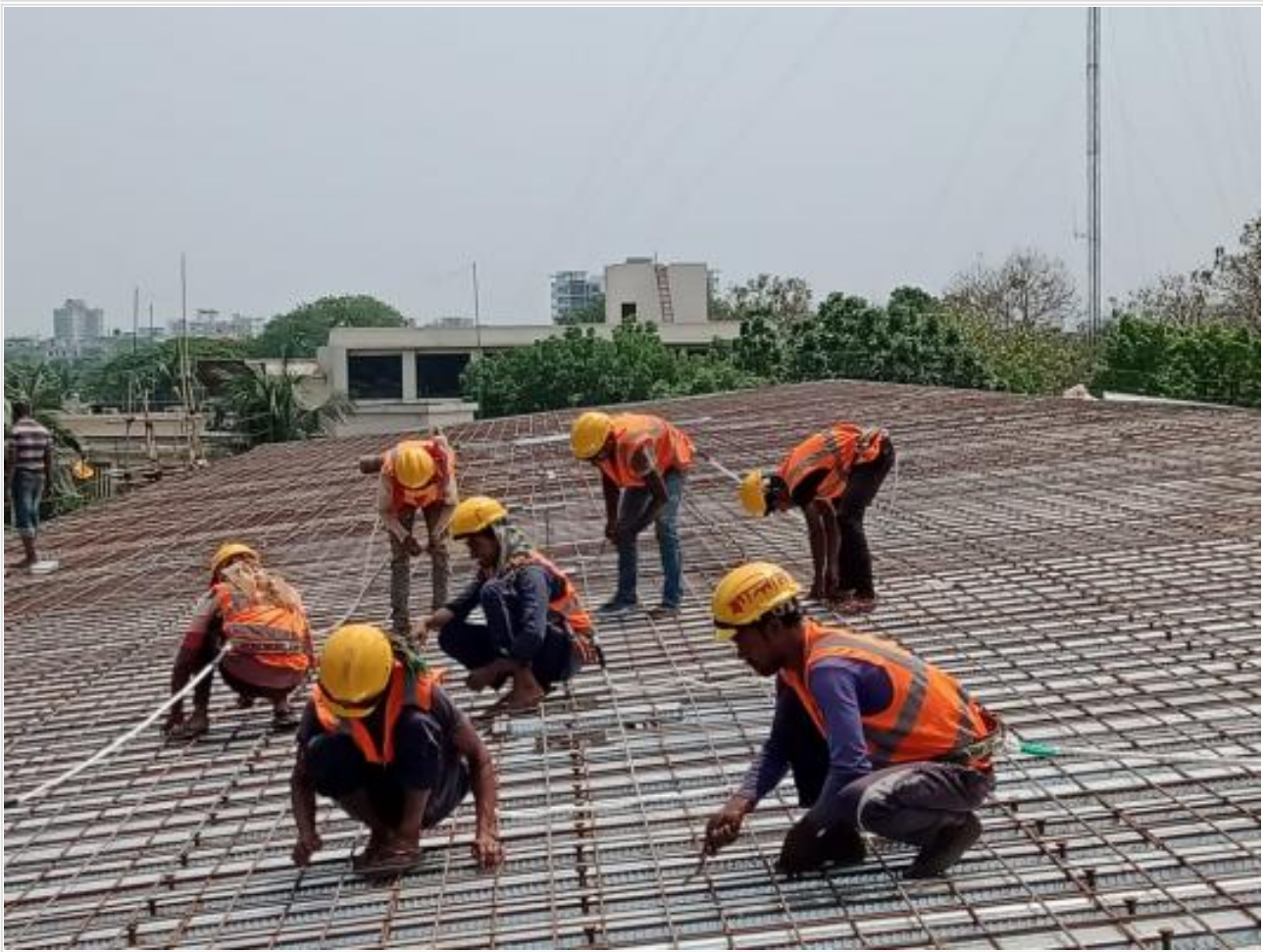
Roof Slab Re-bar Work on 01-05-21
