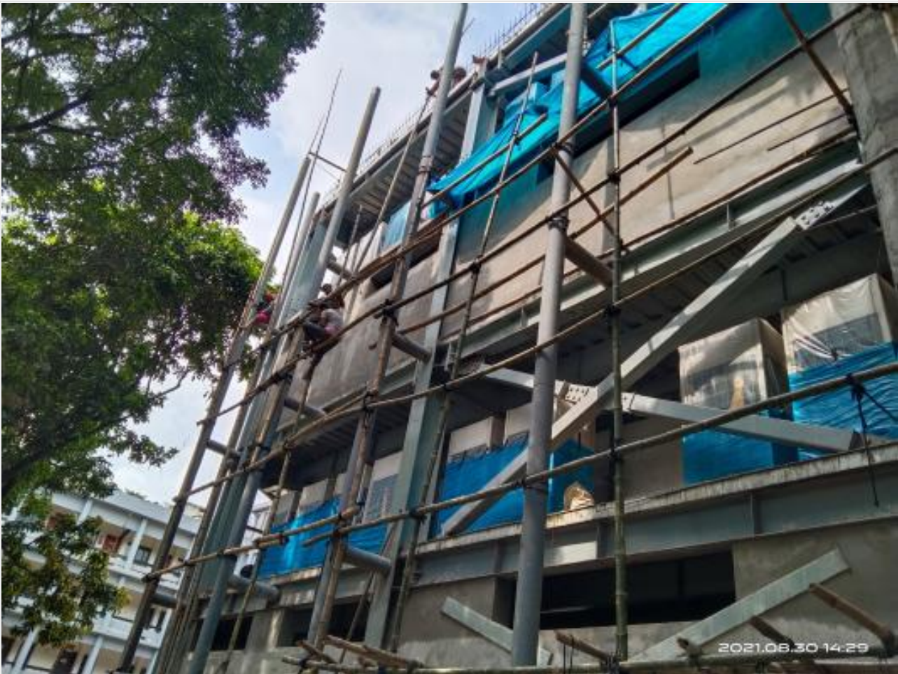
Gutter Scaffolding work on 30-08-21
