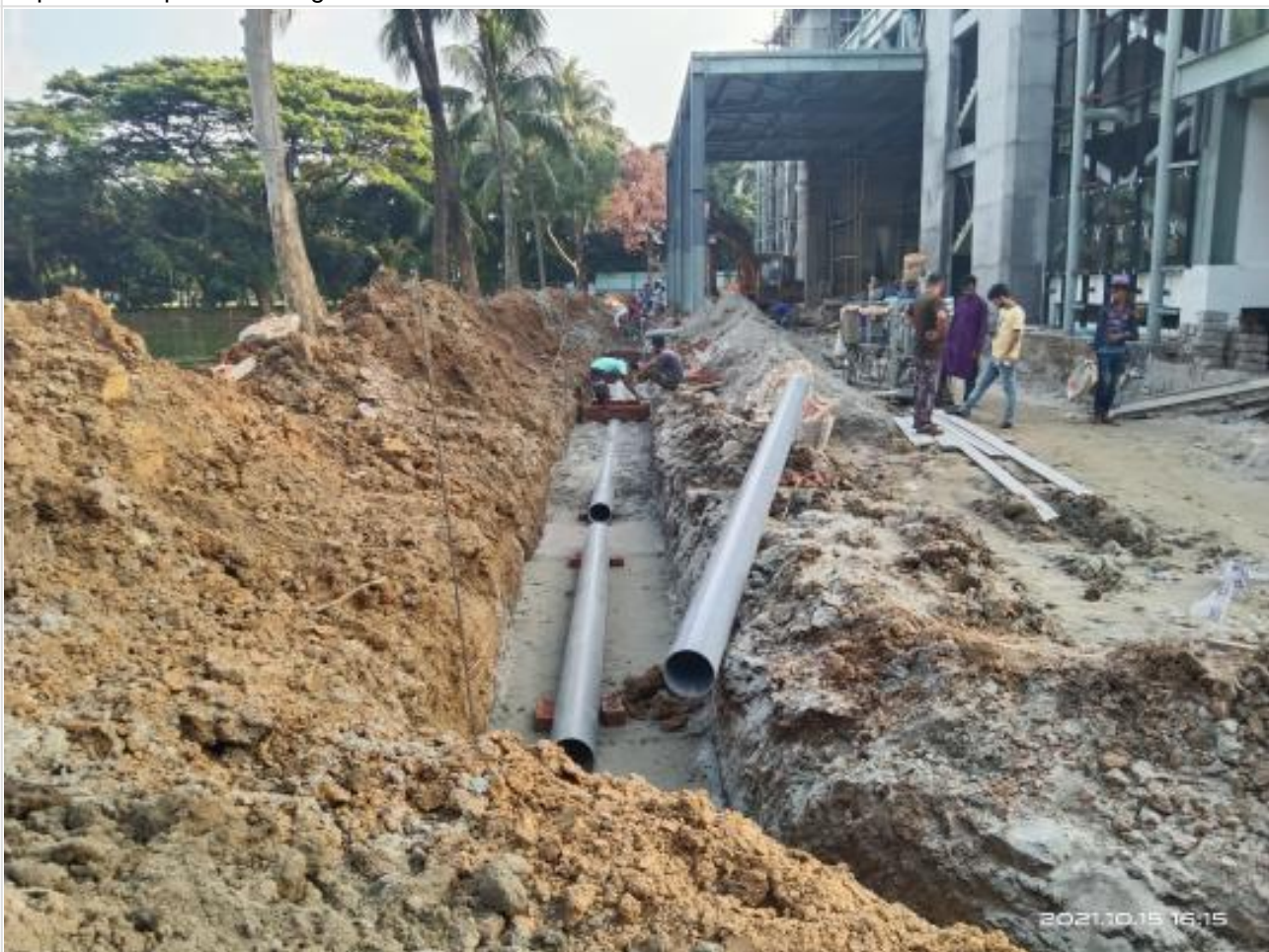
Under ground uPVC pipe line work on 15-10-21
