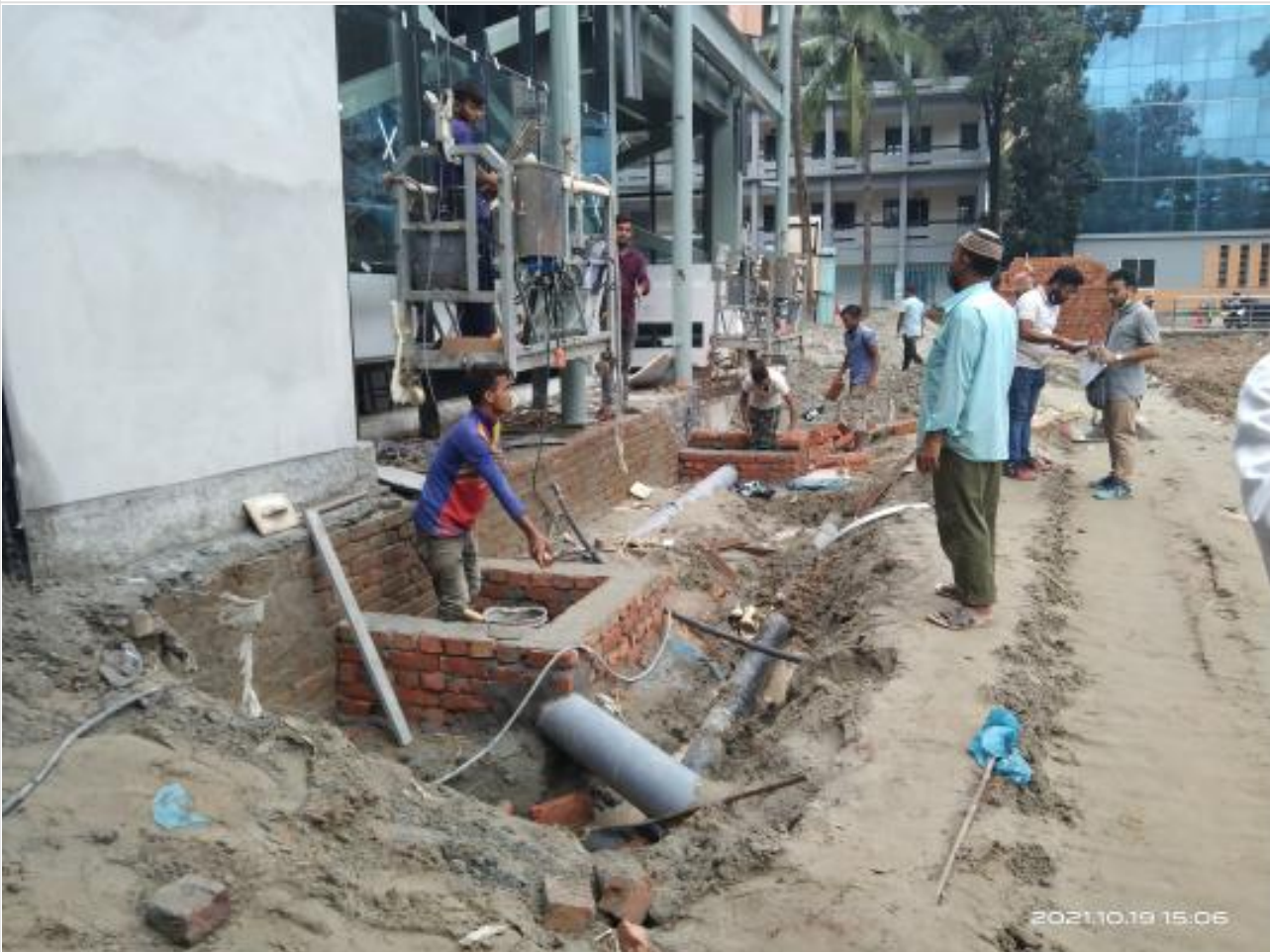
Inspection pit work on 19-10-21
