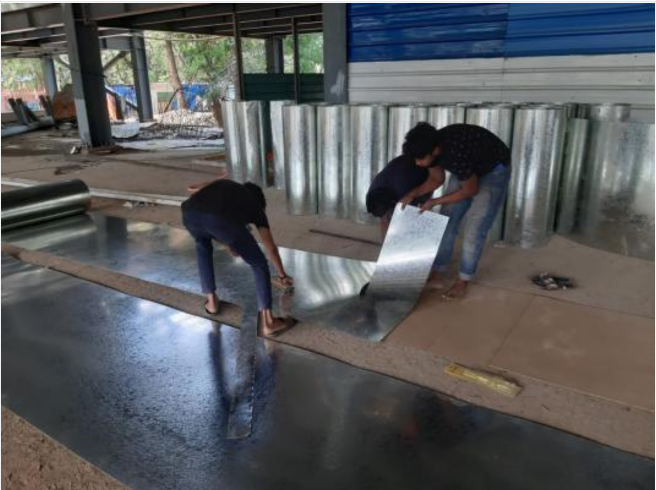
AC Duct Making on 09-05-21
