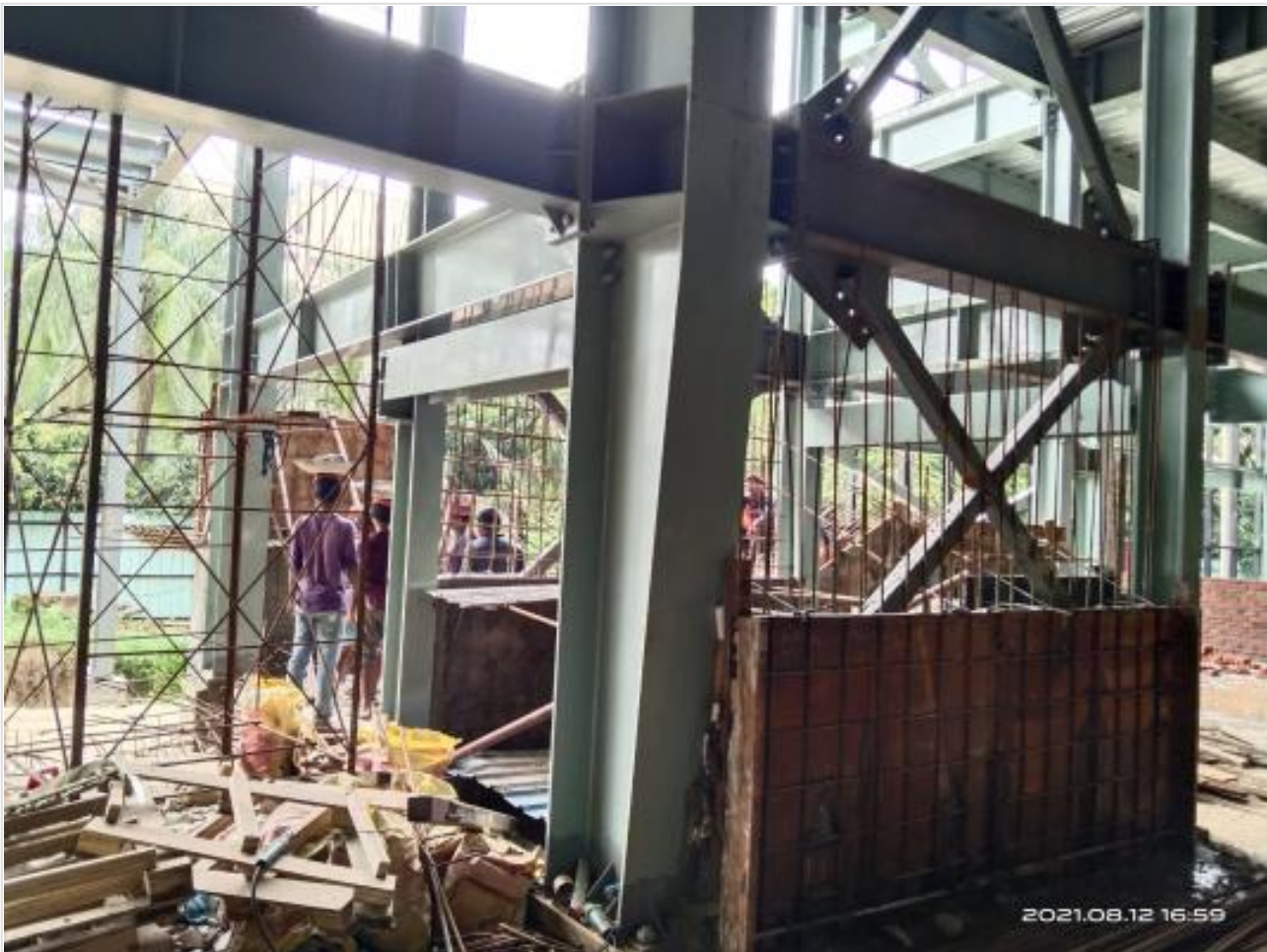
GF Stair work on 12-08-21
