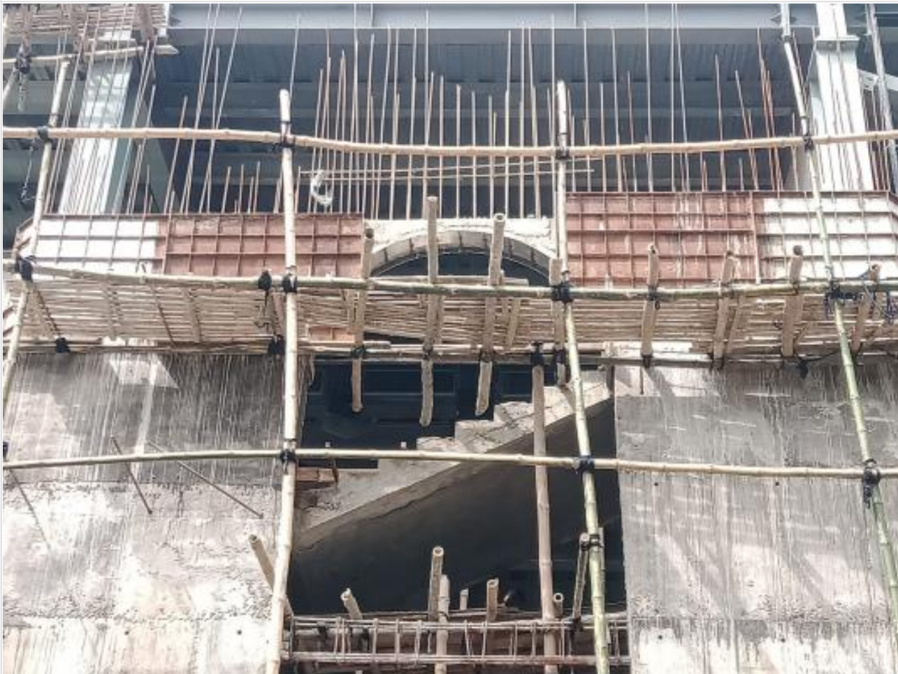
Stair Arch Casting (stair no. 2) on 17-09-21
