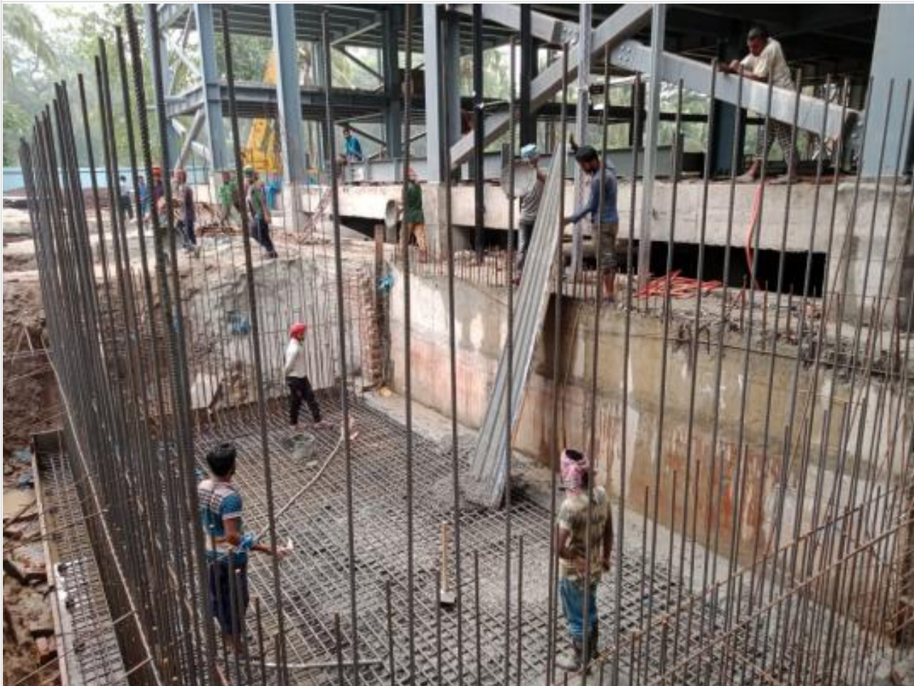
Domestic Water Tank Base concreting on 03-05-21
