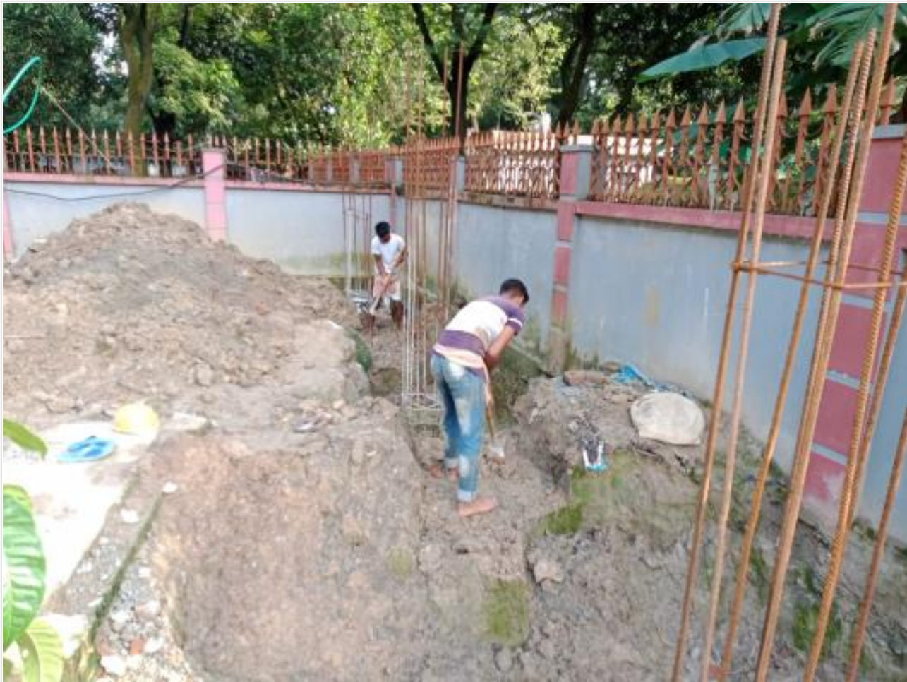
Sub-station grade beam earth cutting on 01-08-21
