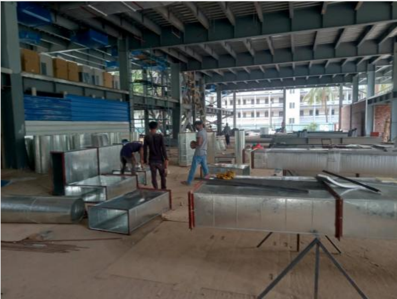
AC Duct Fabrication on 25-05-21
