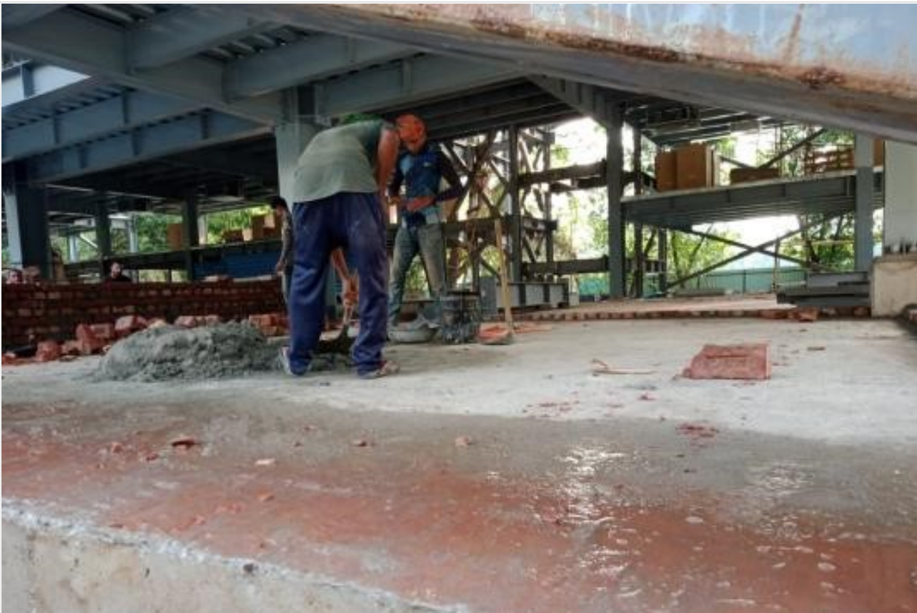
Ground Floor Brick Work on 05-05-21
