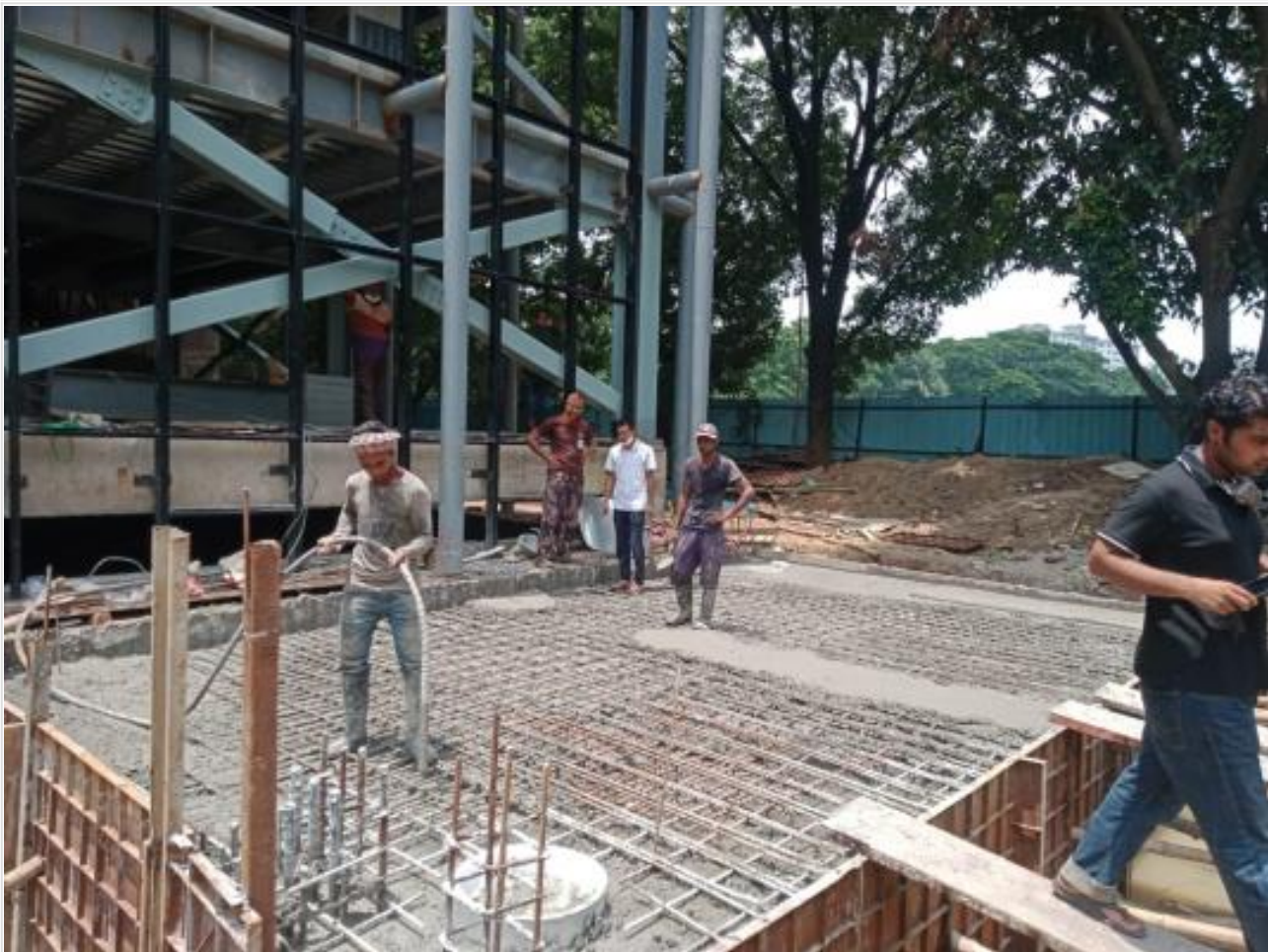
Domestic Water Tank Slab Concreting on 25-06-21
