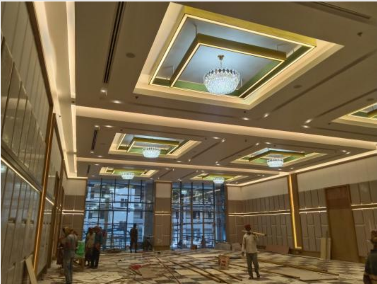
False Ceiling on 16-12-21
