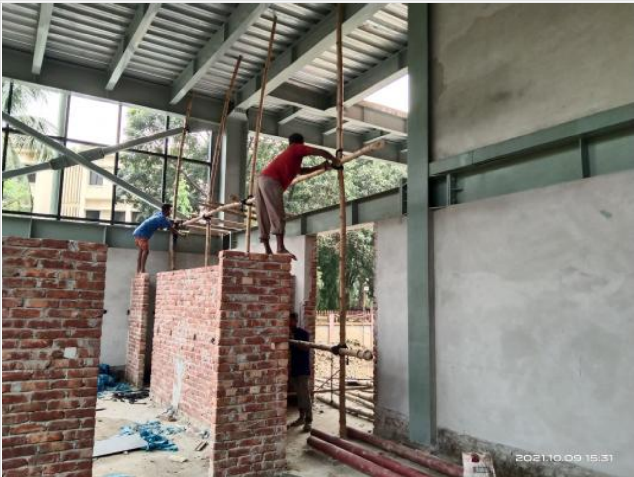
Scaffolding work for brick wall on 09-10-21
