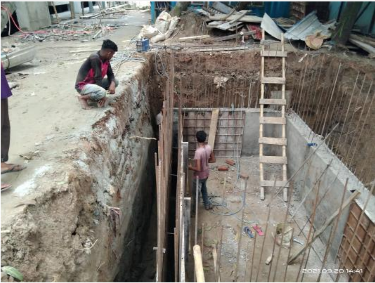
Septic Tank wall shuttering and casting on 20-09-21
