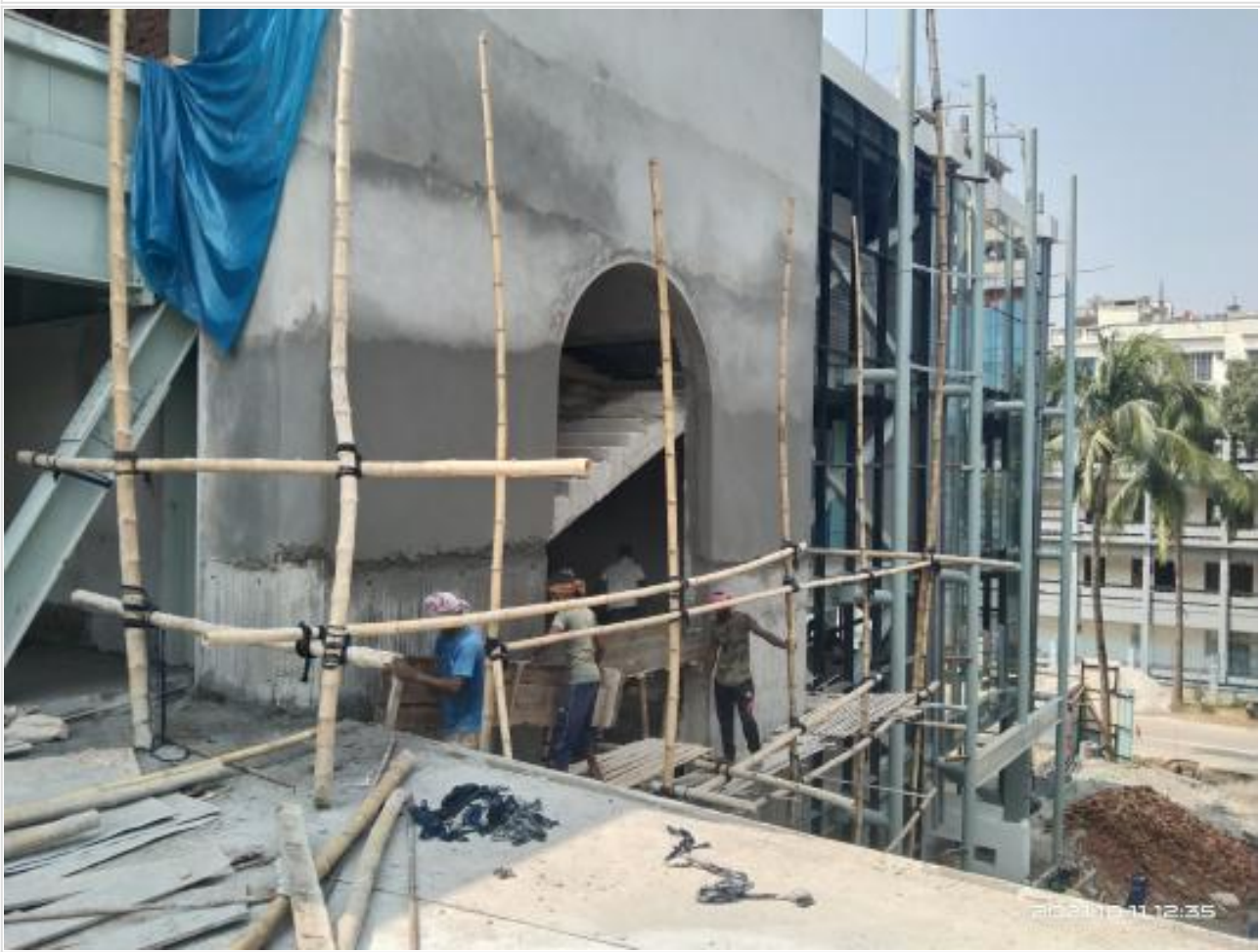
Stair no.2 Outside plaster on 11-10-21
