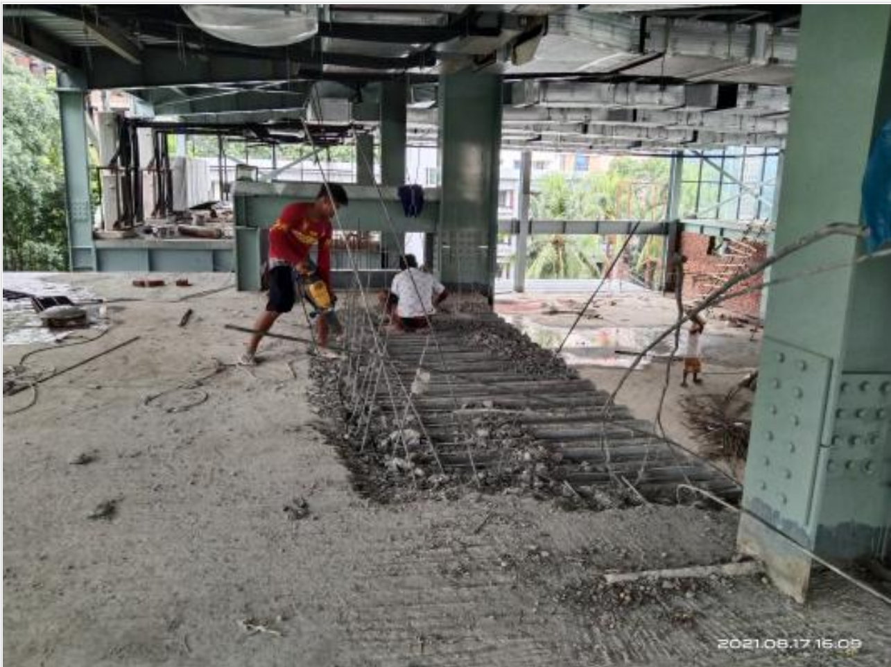
FF Mezzanine slab dismantling on 17-08-21
