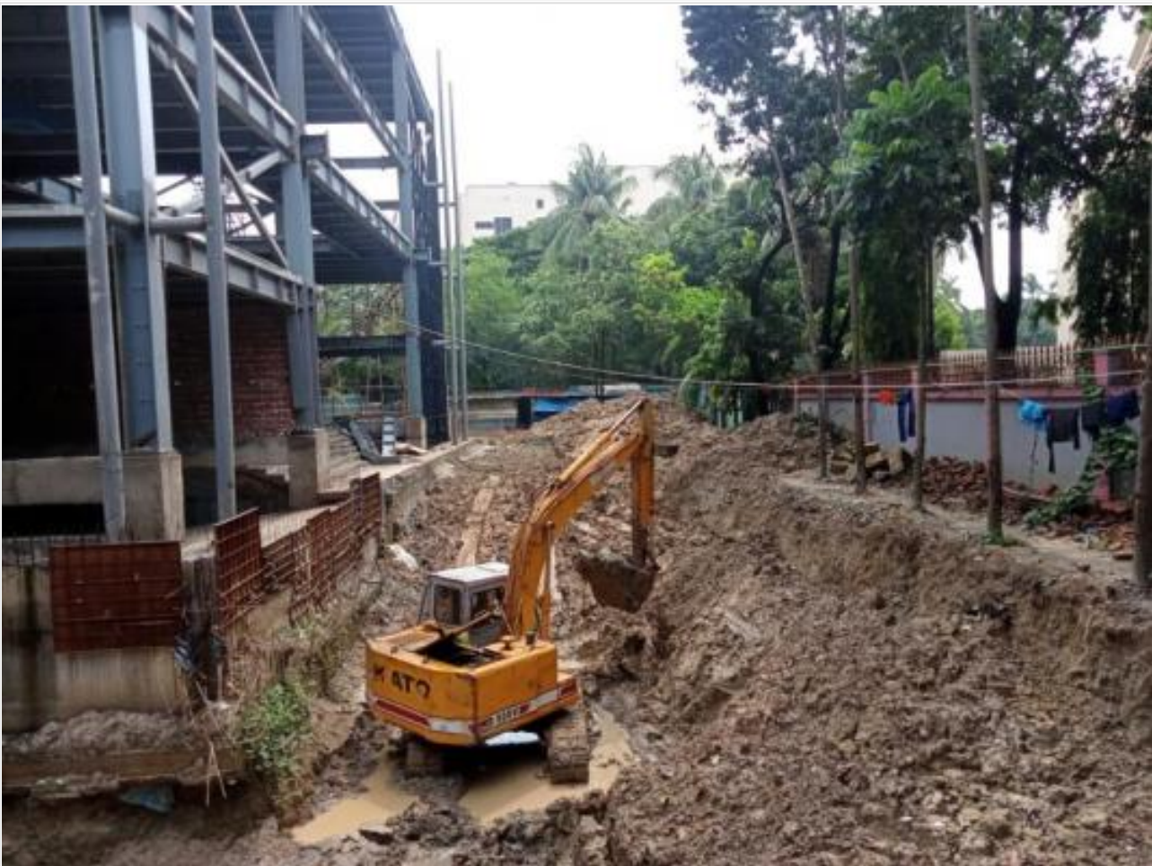
Fire water reservoir excavation on 07-06-21
