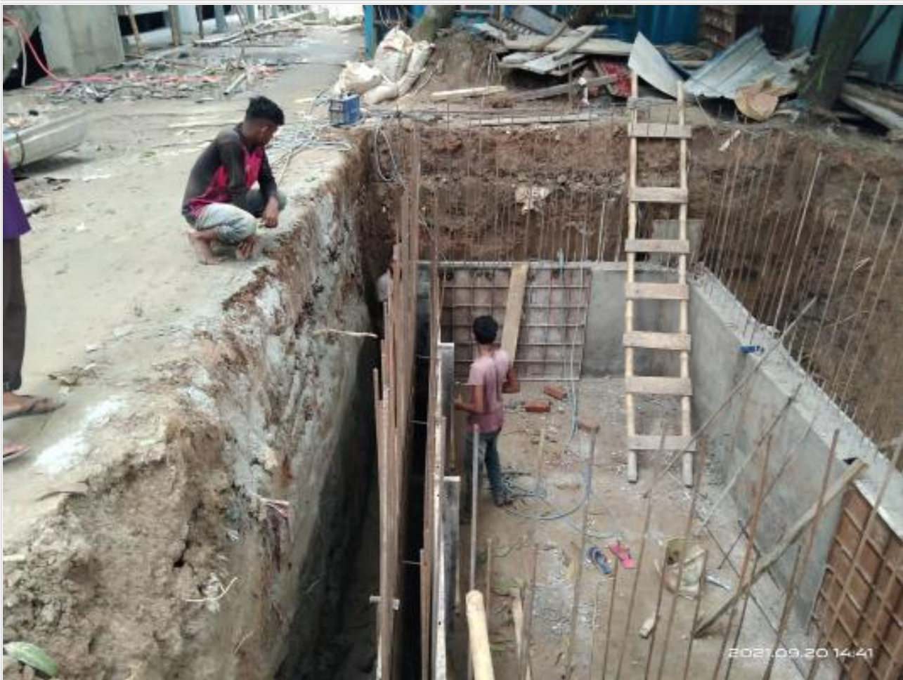
Septic Tank wall shuttering and casting on 20-09-21
