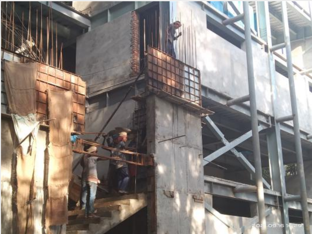
Stair wall casting on 16-09-21
