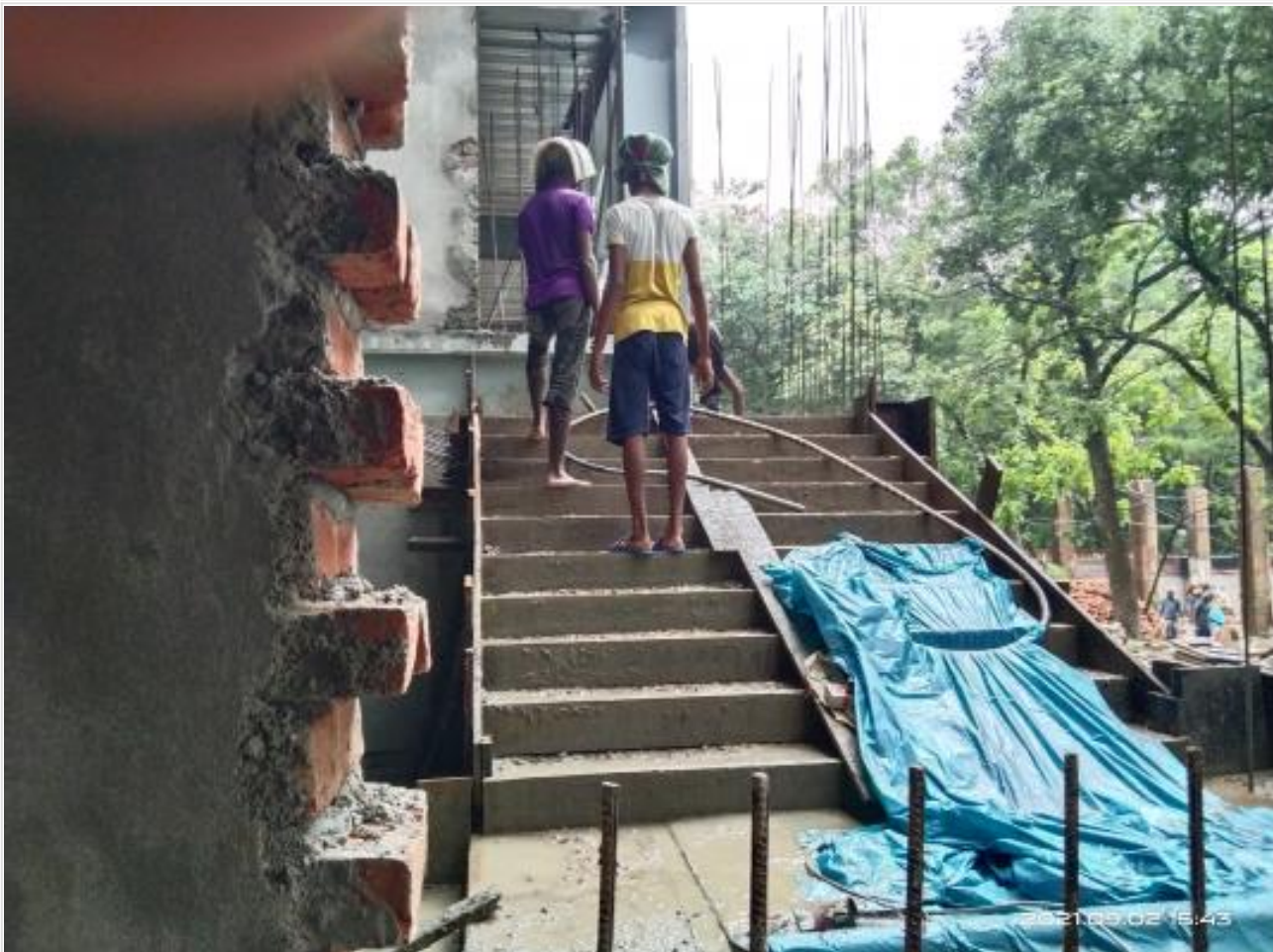
Grond floor stair casting on 02-09-21
