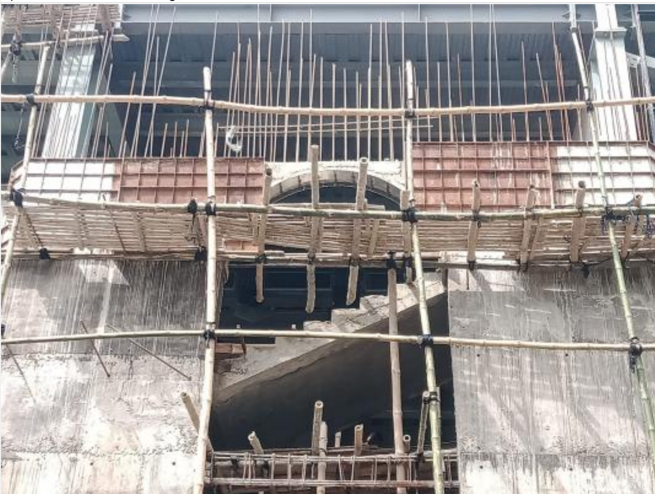
Stair Arch Casting (stair no. 2) on 17-09-21
