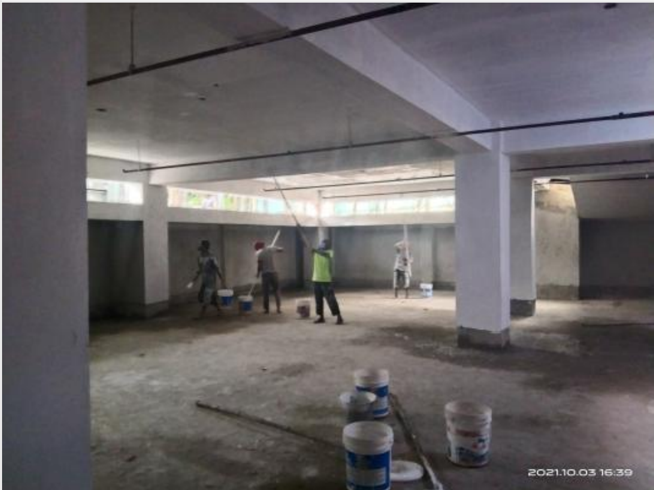
Basement wall and ceiling paint on 03-10-21
