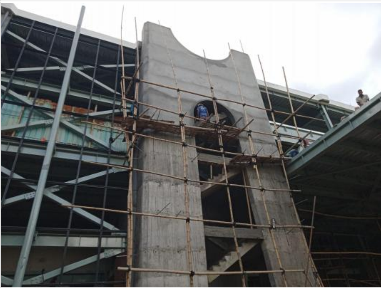
Outside stair plaster on 18-10-21
