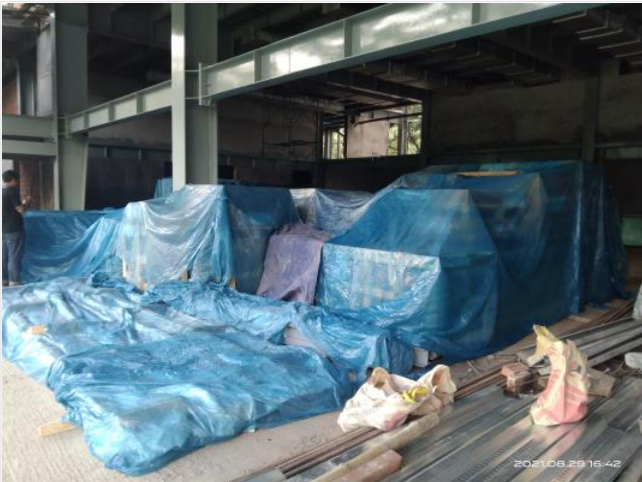
Lift receive at site on 29-08-21
