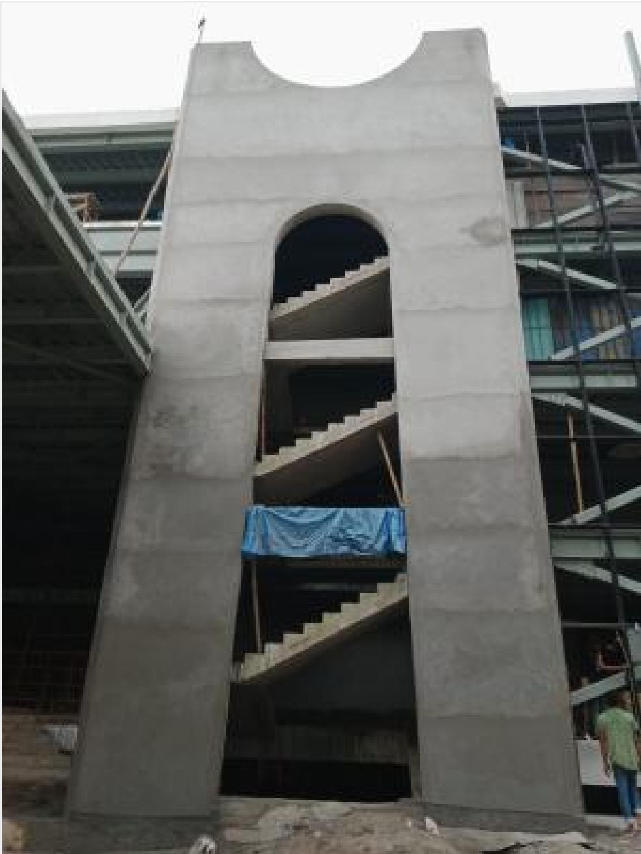
Stair-02 outside plaster complete on 14-10-21
