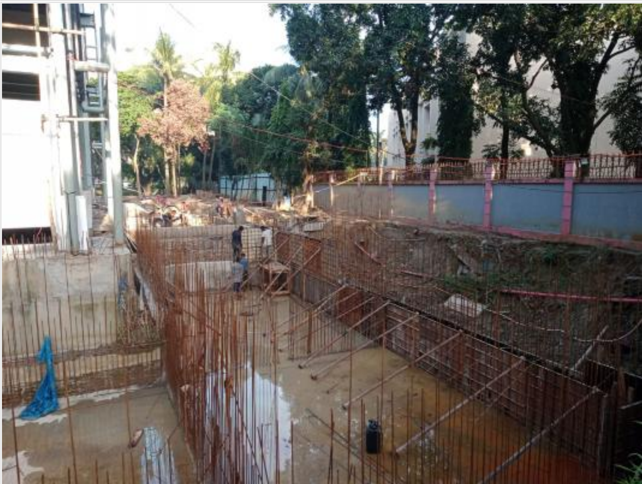
Fire Tank wall shuttering on 17-10-21
