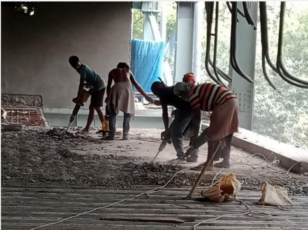
FFM slab dismantling work on 27-08-21
