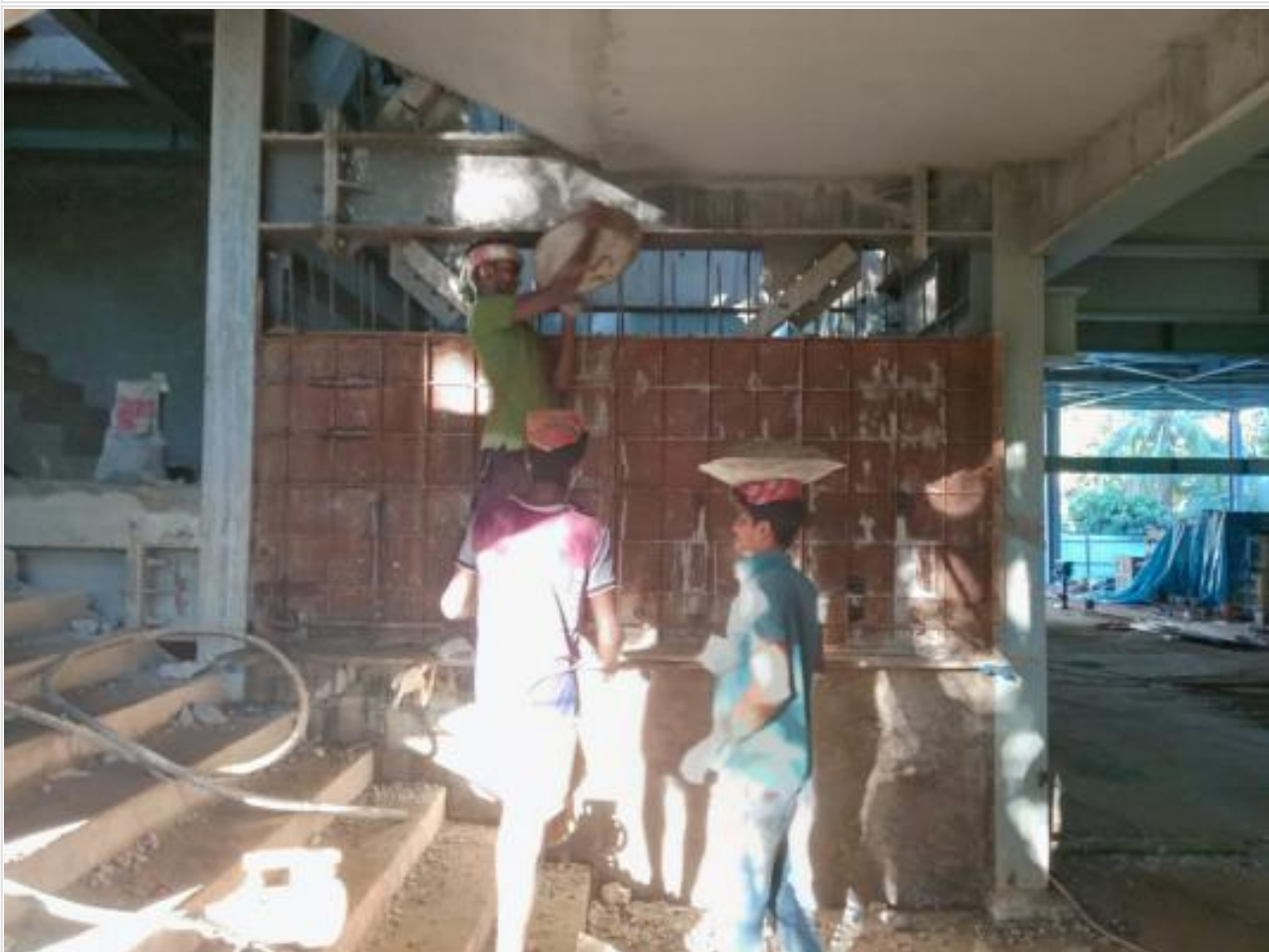
GF Lift wall Casting on 31-08-21
