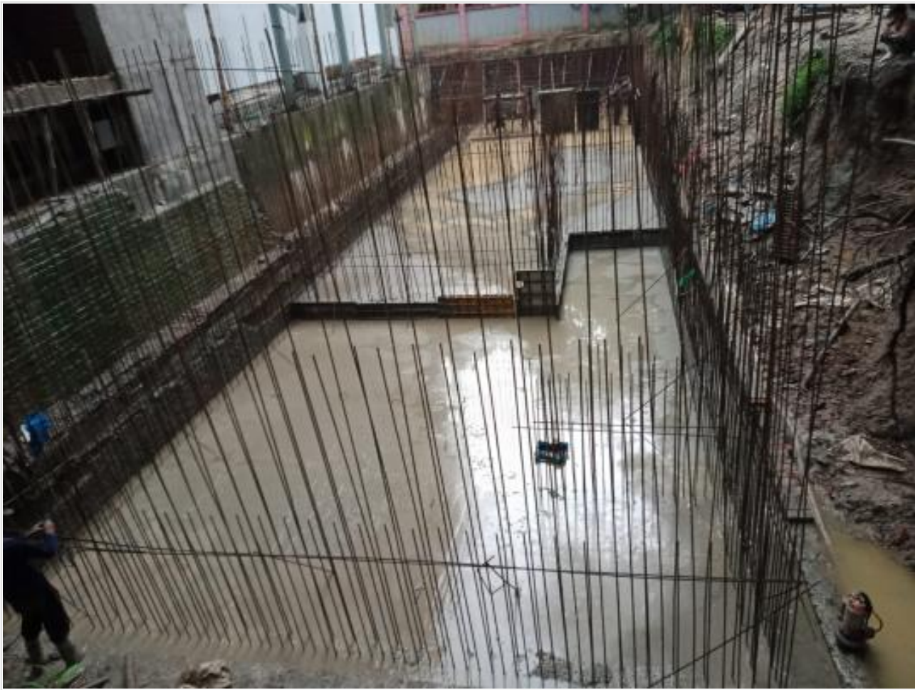
Fire Tank base casting on 20-10-21
