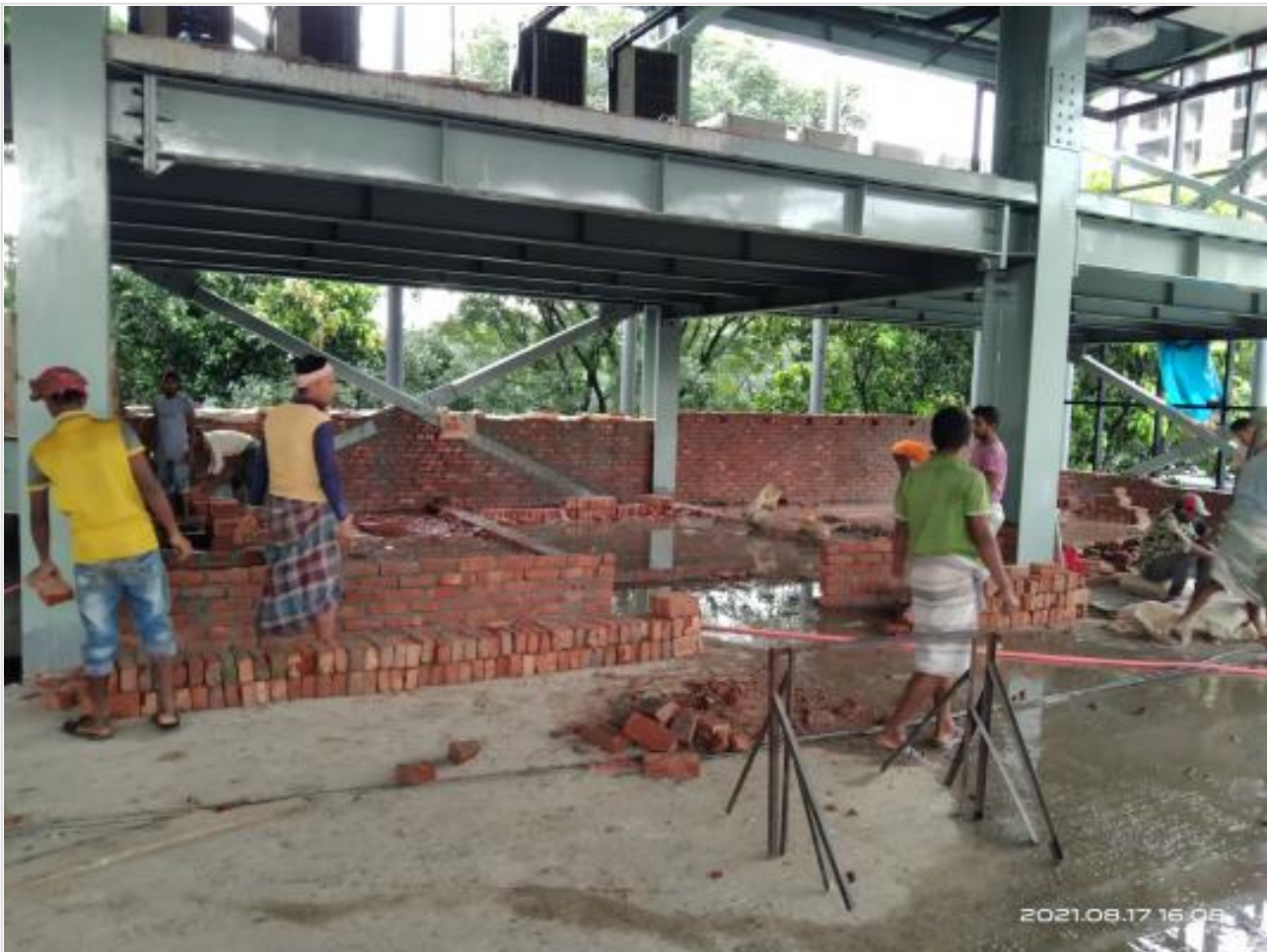
GF brick work on 17-08-21
