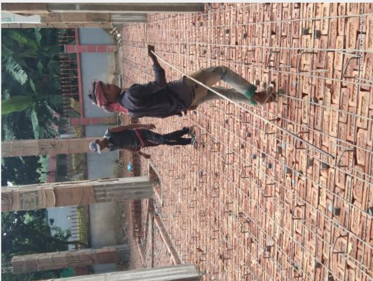
Generator floor rod binding on 05-09-21
