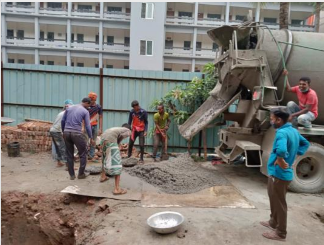
Canopy Base Concreting on 03-05-21
