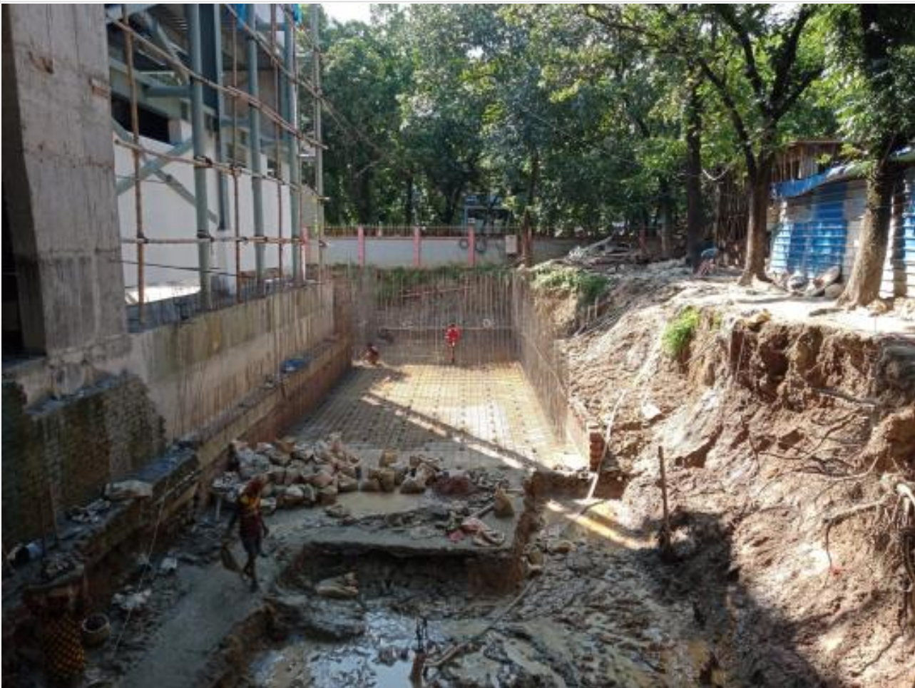
Fire tank base and wall rod binding on 01-10-21
