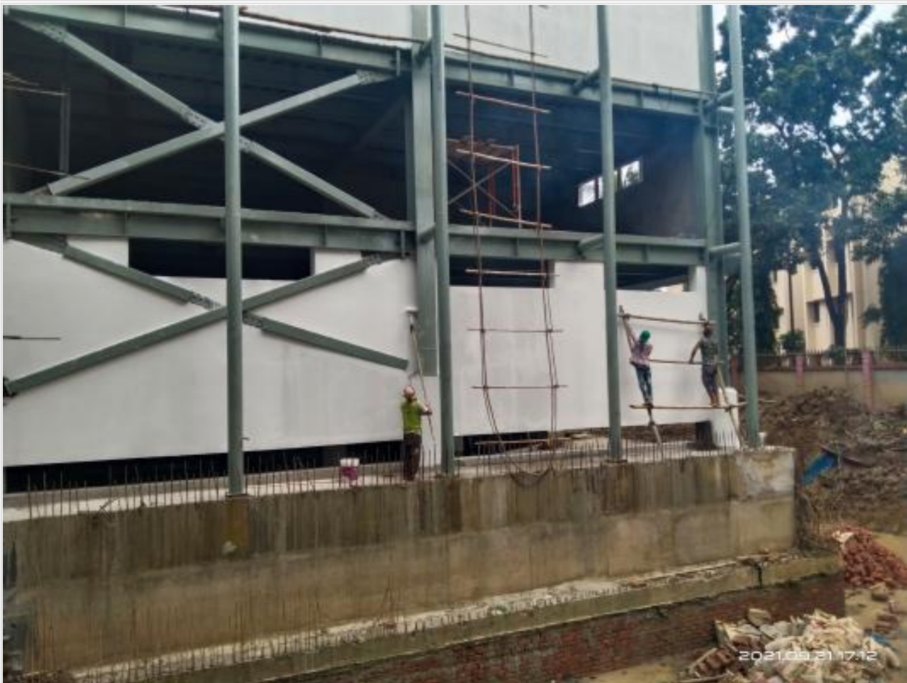
Exterior wall painting work on 21-09-21
