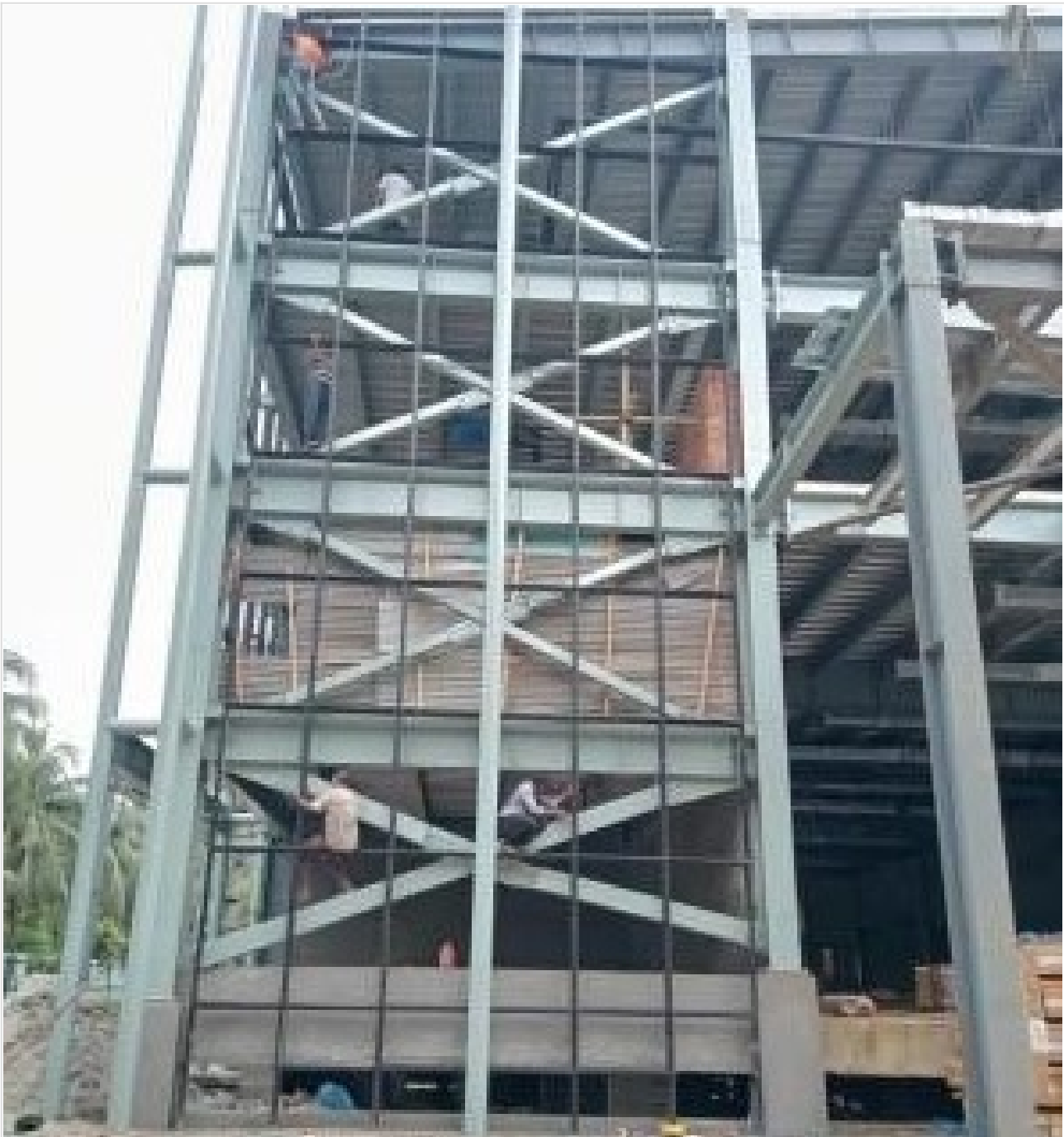
Out side glass frame cleaning on 13-08-21
