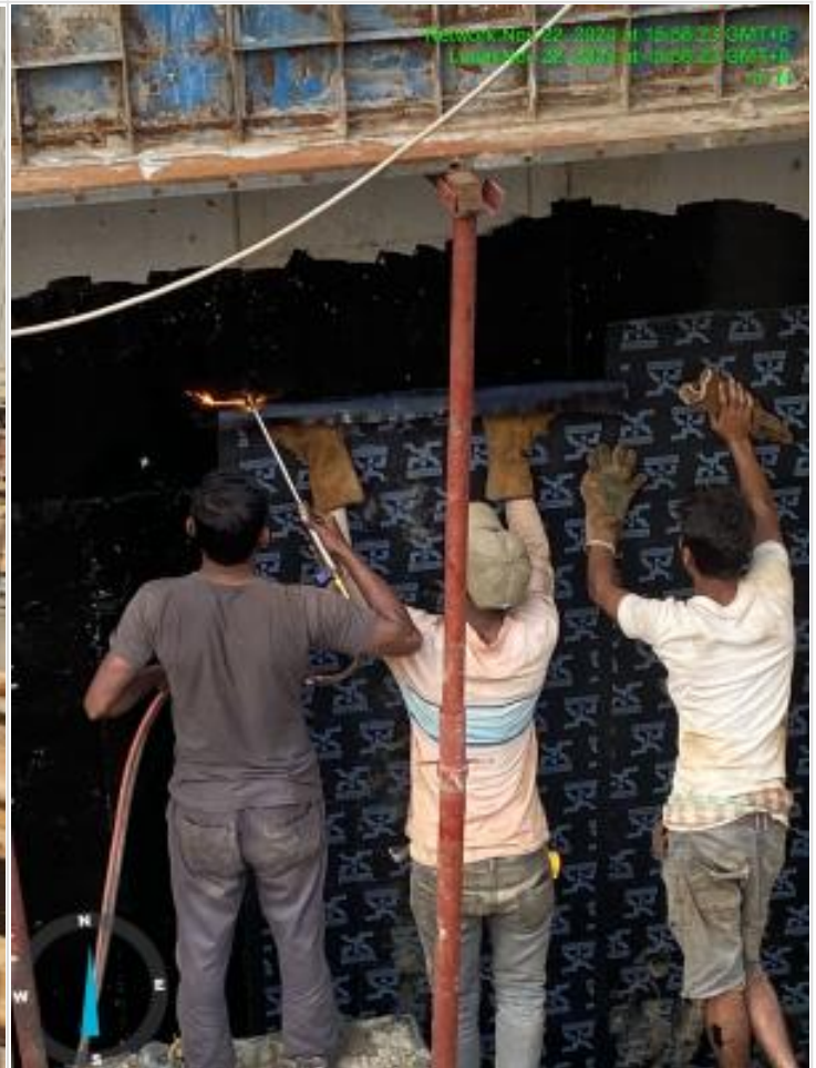
Tank wall water proofing membrain SBS fi
