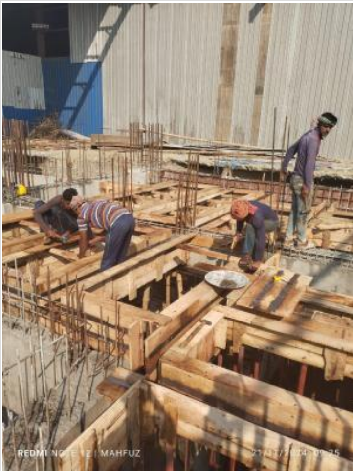
Tank slab shuttering
