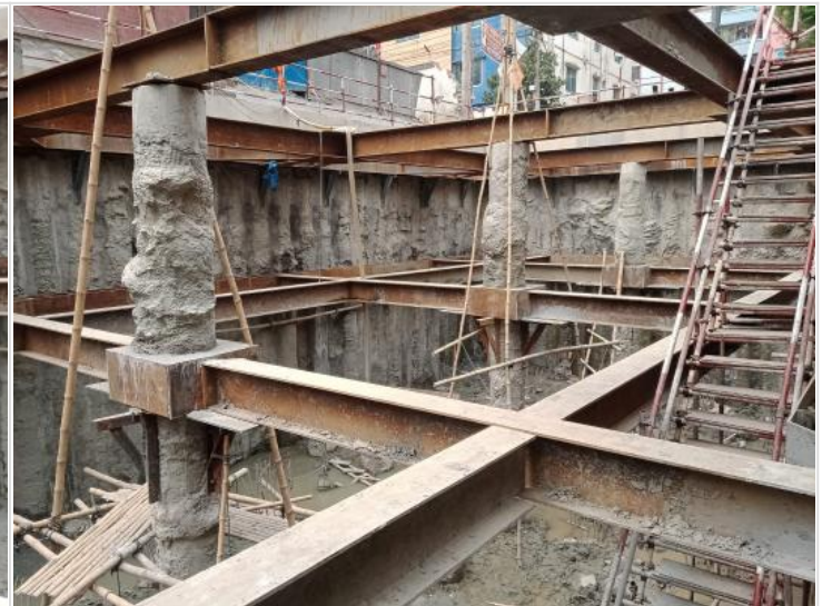
Pile gap water proofing
