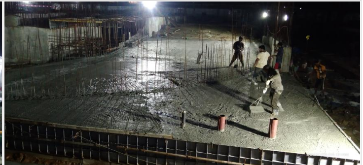
Ready mix concreting
