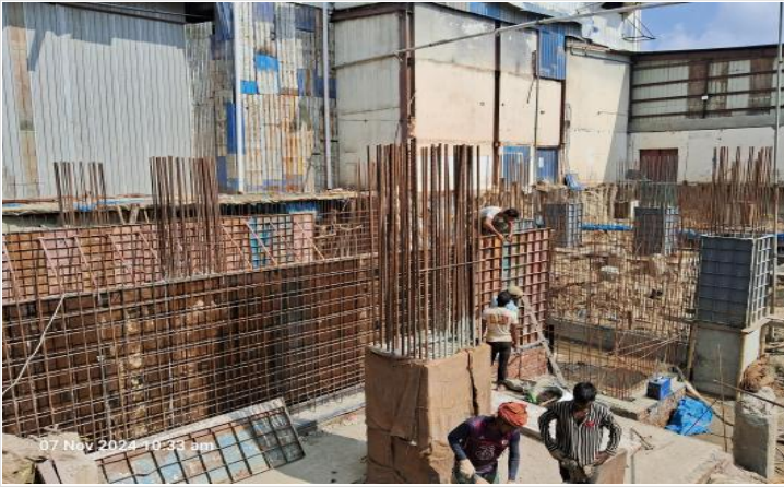
Wall shuttering on 07-11-24
