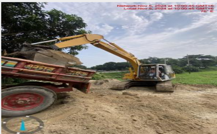
Earth loading for backfilling on 05-11-24
