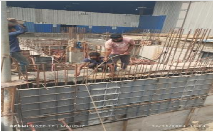
Wall concreting on 16-11-24
