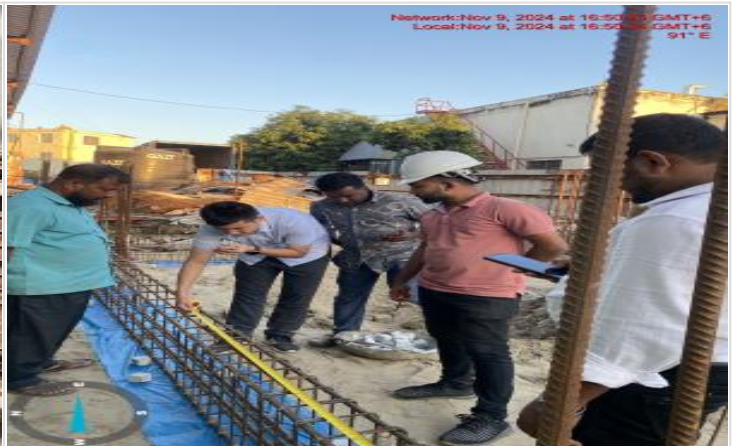
Foundation beam rebar inspection on 09-11-24
