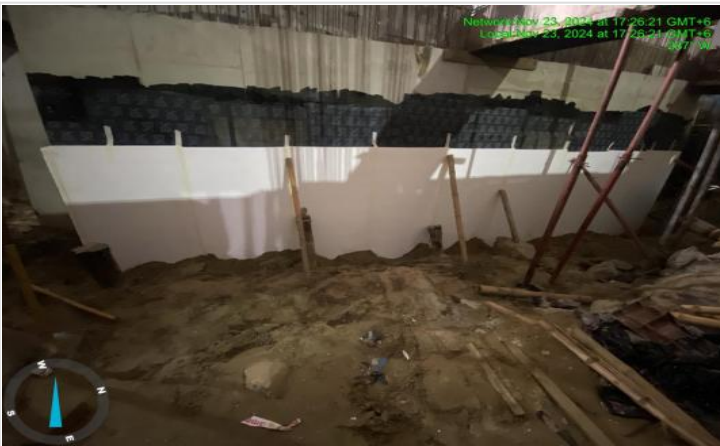
Tank wall stylo foam fixing on 23-11-24
