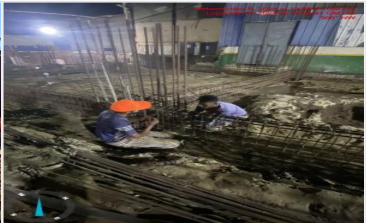
Foundation beam rebar work on 08-11-24
