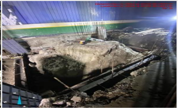
Bracing beam concreting on 02-11-24
