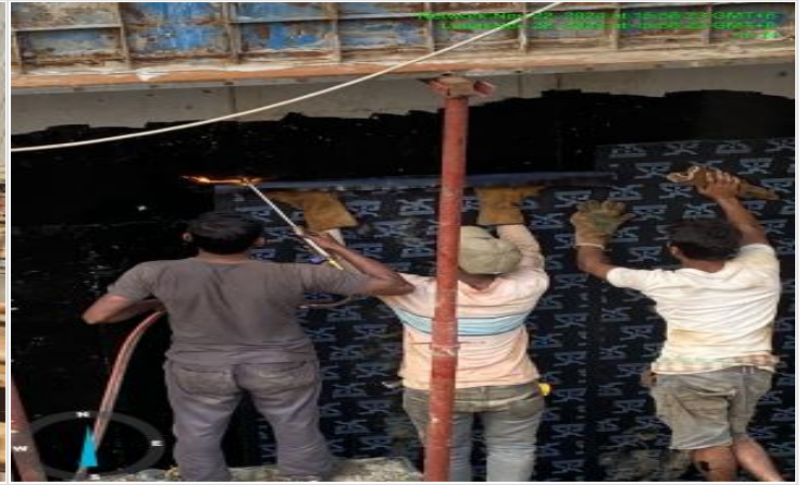
Tank wall water proofing membrain SBS fi on 22-11-24
