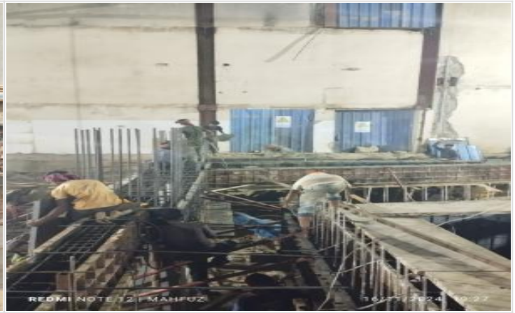
Foundation beam concreting on 16-11-24
