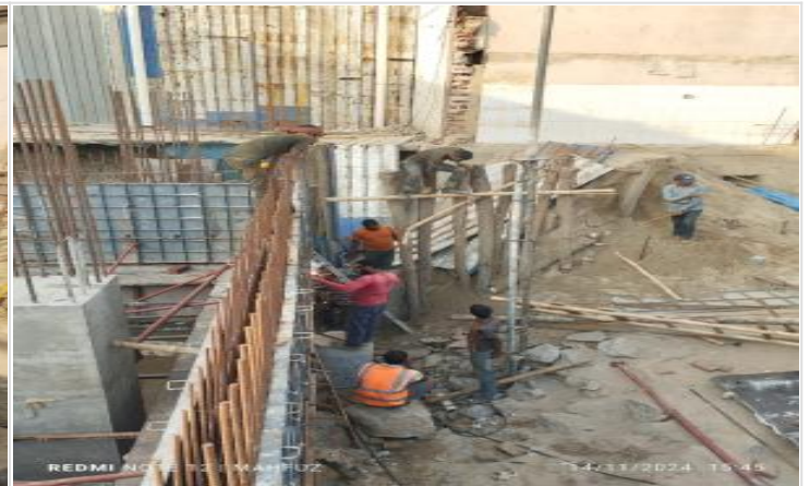
Wall shuttering on 14-11-24
