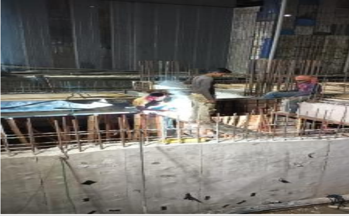
Tank slab shuttering on 21-11-24
