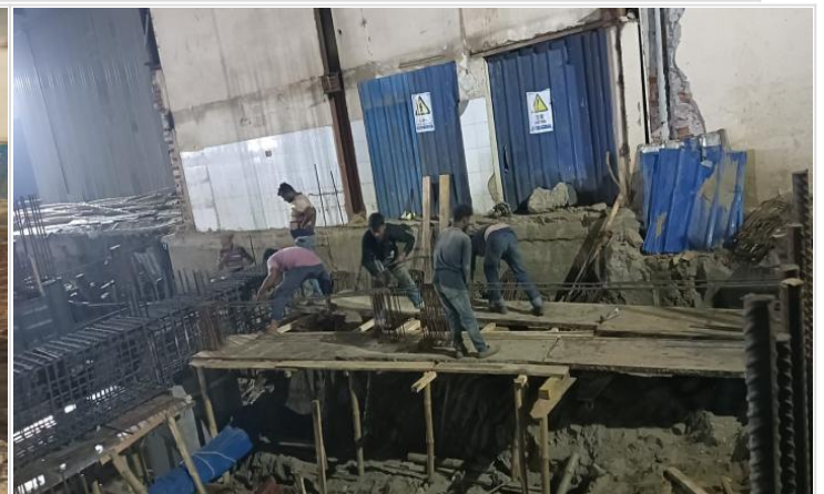
Foundation beam rebar work on 15-11-24
