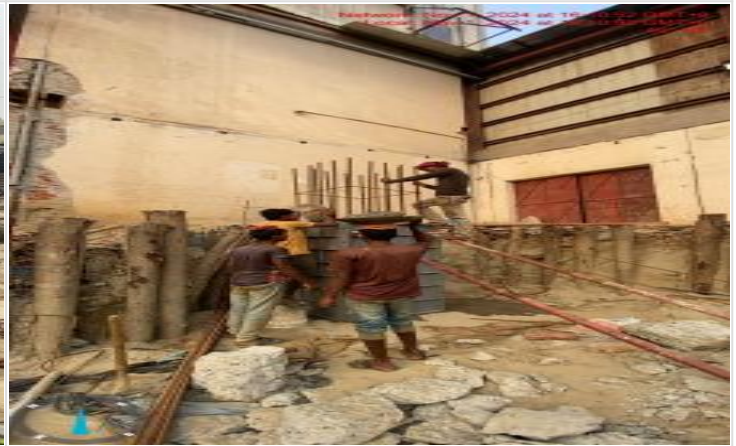
Column concreting on 01-11-24
