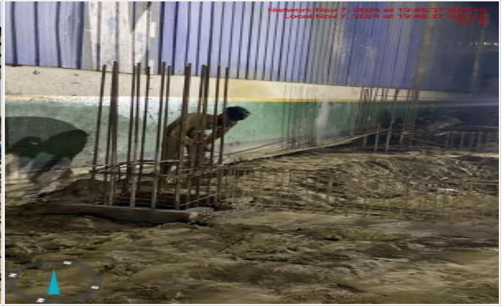
Column re-bar work on 07-11-24
