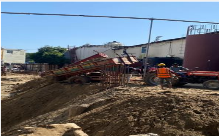
Backfilling on 08-11-24
