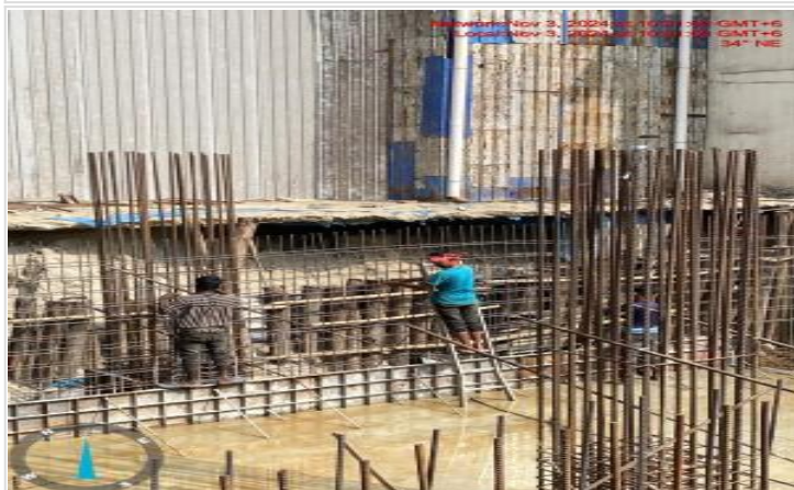
Wall re-bar work on 03-11-24
