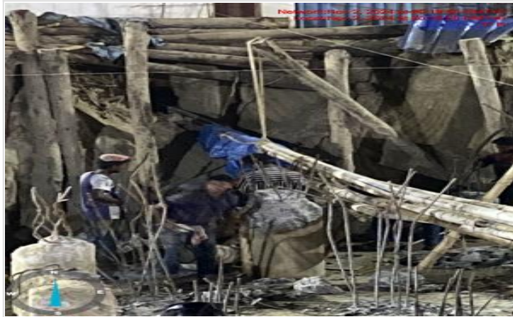
Pile head breaking on 02-11-24
