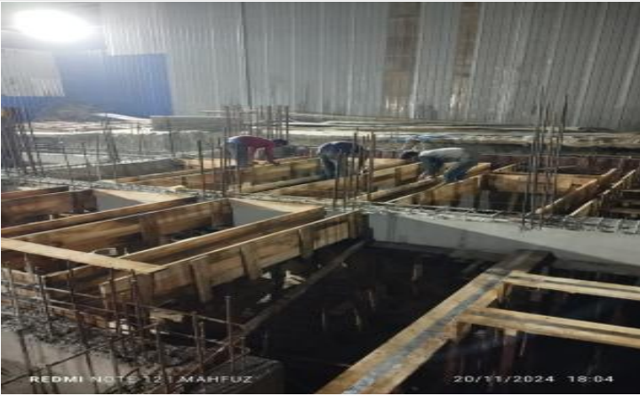
Tank slab shuttering on 20-11-24
