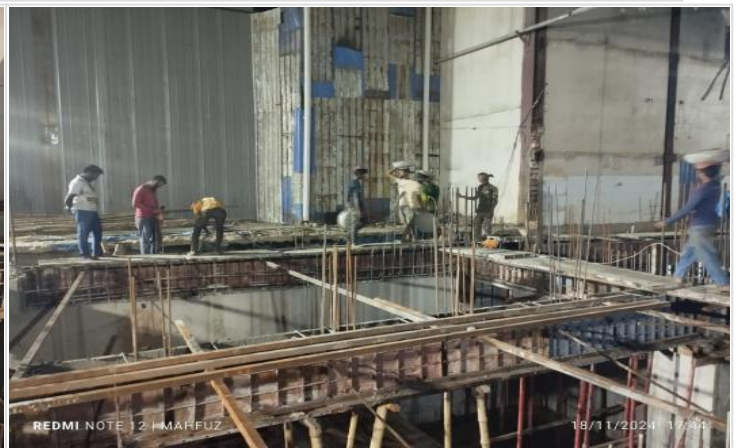
Foundation beam concreting on 18-11-24
