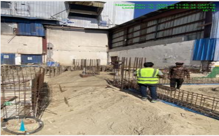
Foundation beam rebar work on 10-11-24
