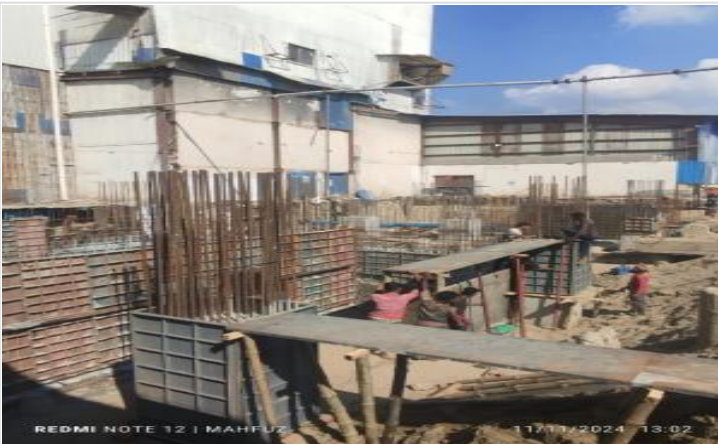
Foundation beam shuttering on 11-11-24
