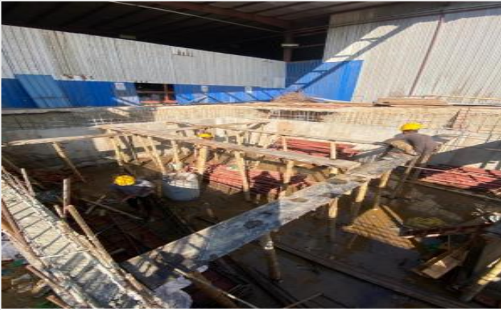
Tank slab shuttering on 20-11-24
