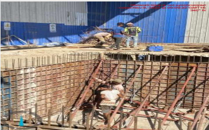
Wall shuttering on 09-11-24
