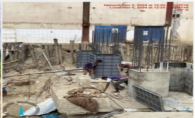
Column shuttering on 05-11-24
