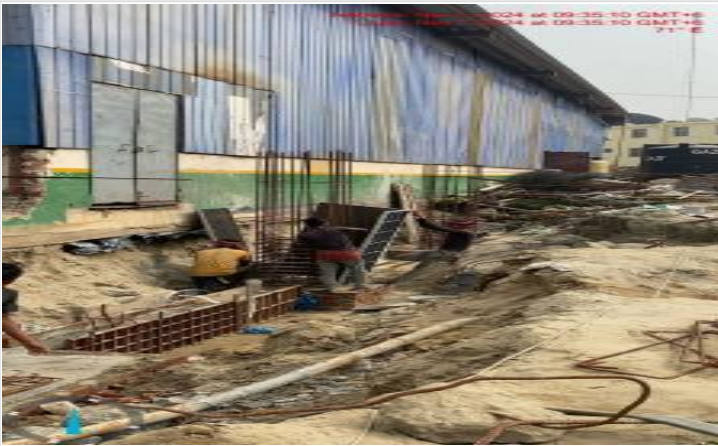
Bracing beam- Column shuttering on 01-11-24
