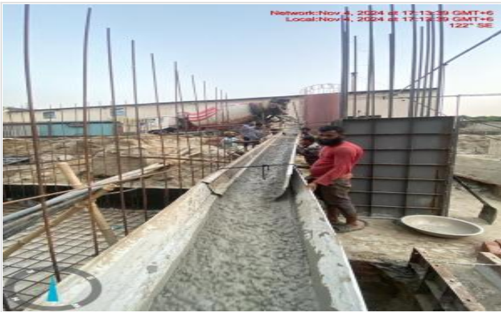
Pile cap Concreting on 04-11-24
