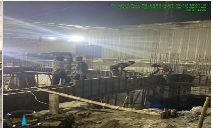
Foundation beam concreting on 12-11-24
