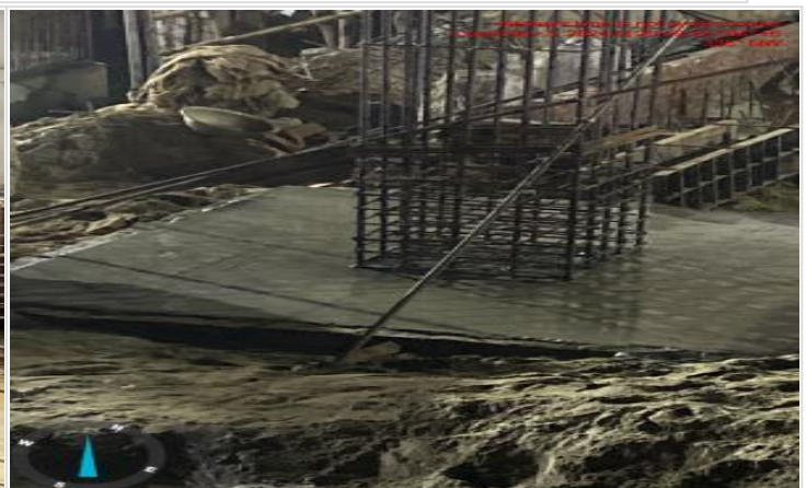
Pile cap concreting on 03-11-24
