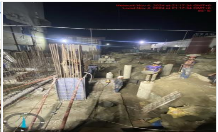
Column concreting on 04-11-24
