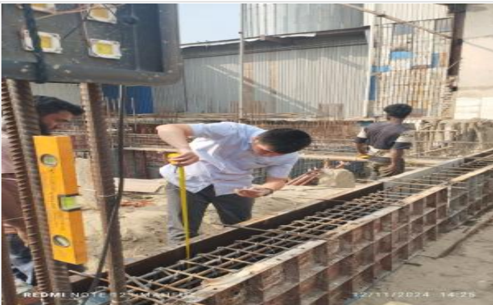
Foundation beam inspection before concrete on 12-11-24
