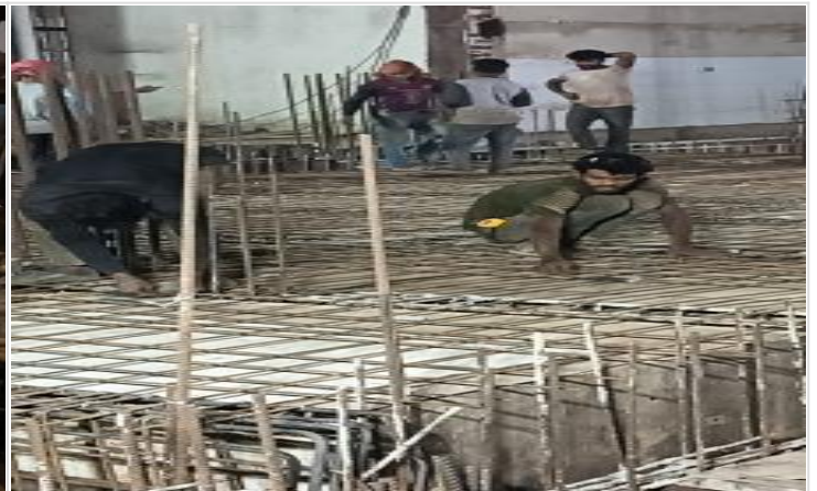
Tank slab re-bar fixing on 23-11-24
