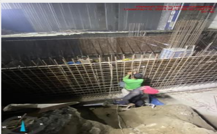
Wall shuttering on 06-11-24
