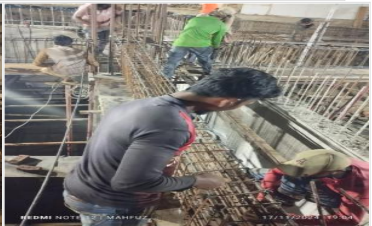
Foundation beam rebar work on 17-11-24
