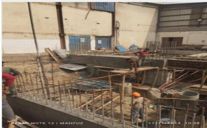
Foundation beam bottom shuttering on 17-11-24
