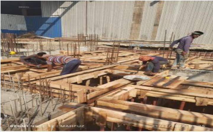
Tank slab shuttering on 22-11-24
