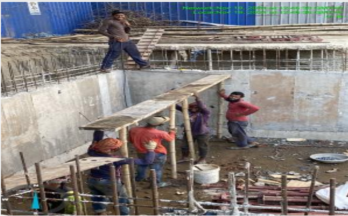
Tank slab shuttering on 19-11-24
