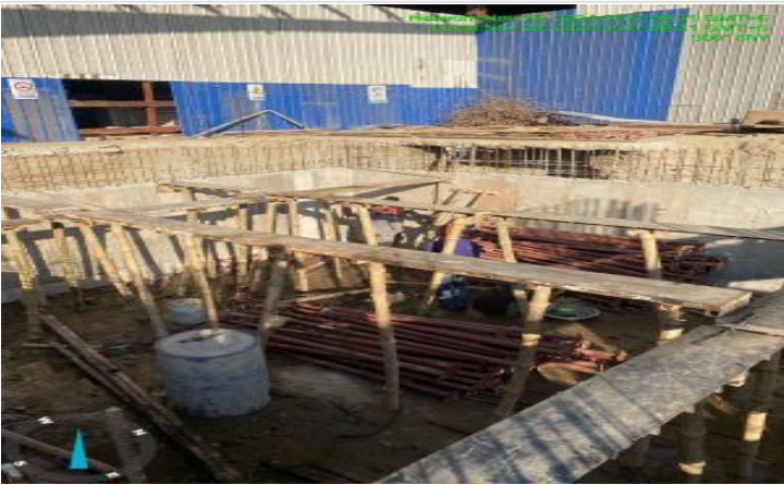
Tank slab shuttering on 19-11-24
