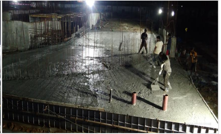
Ready mix concreting on 03-06-22
