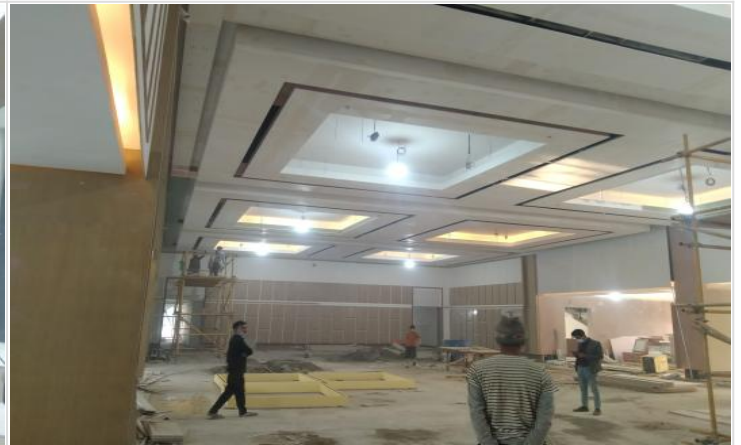
Interior work on 31-01-22
