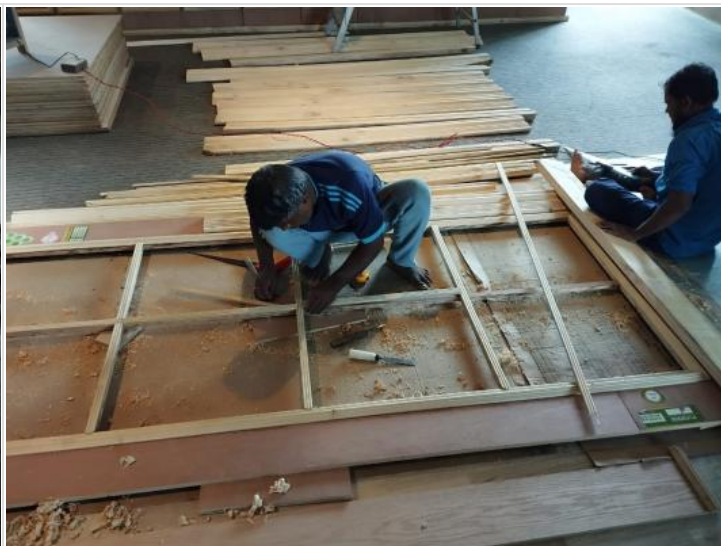
11th Floor Interior Work
