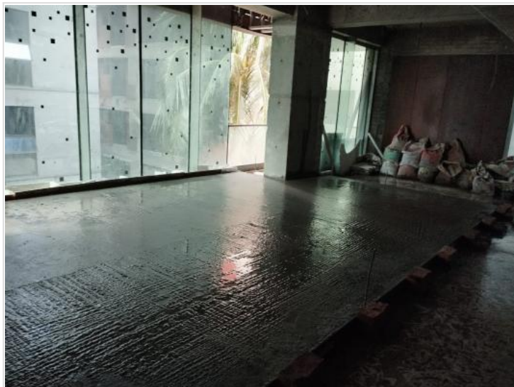
4th Flr-Floor Raining Concreting Complet
