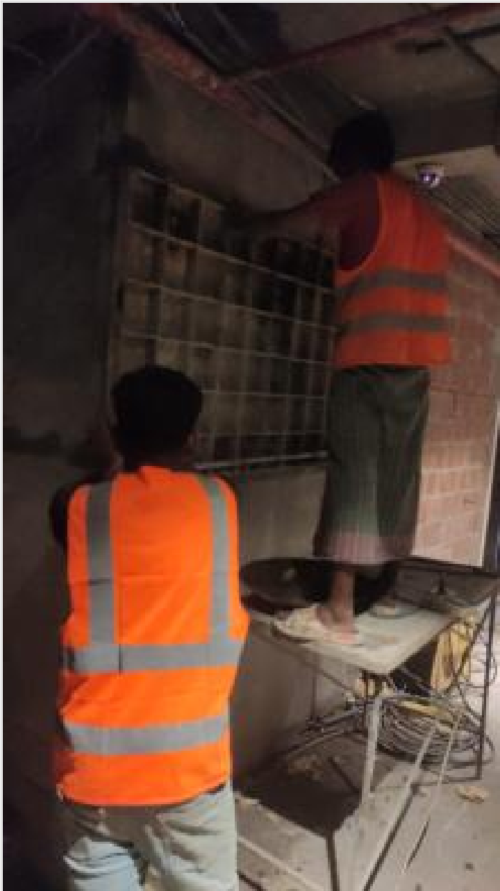
B2-Column Retrofit-Shutter removing
