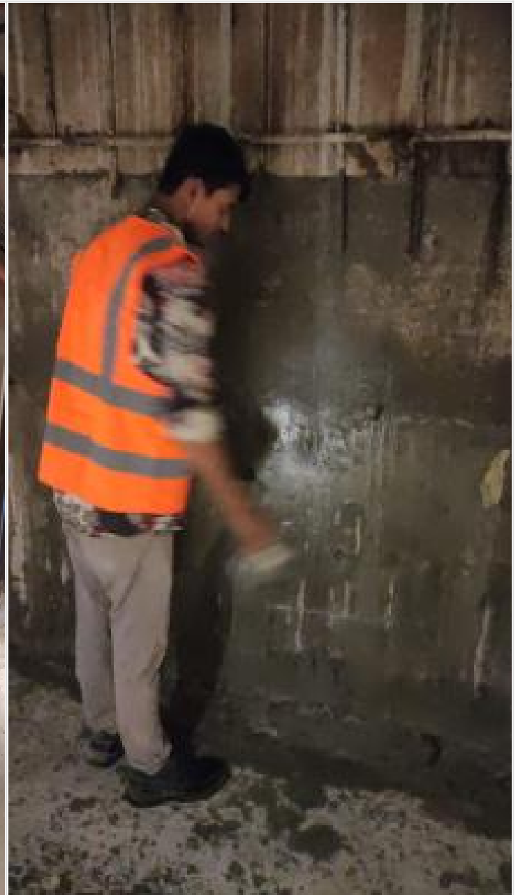
B2-Column Retrofit-Curing
