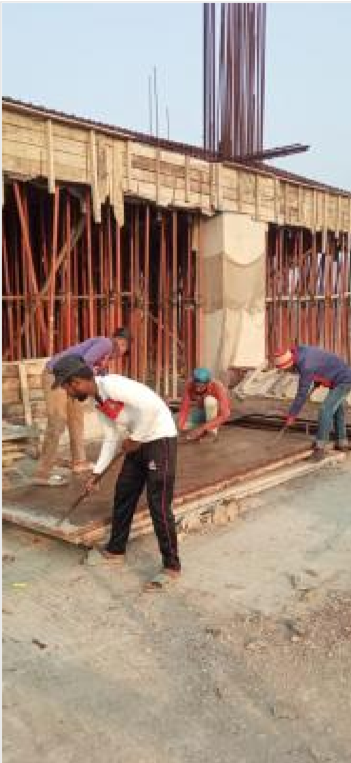
Column/Wall Steel Shutter Cleaning, Oili
