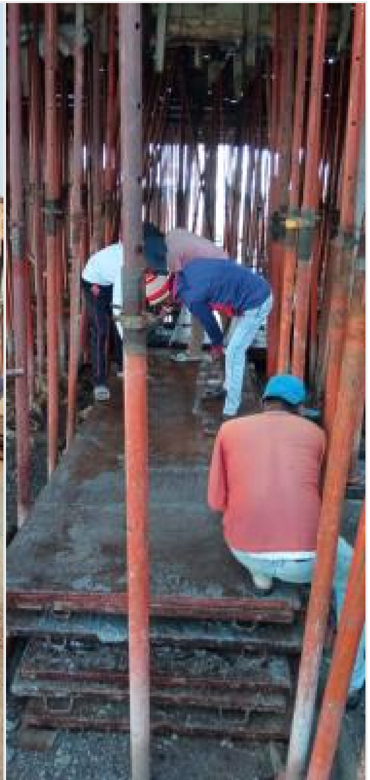
Column/Wall Steel Shutter Cleaning, Oili
