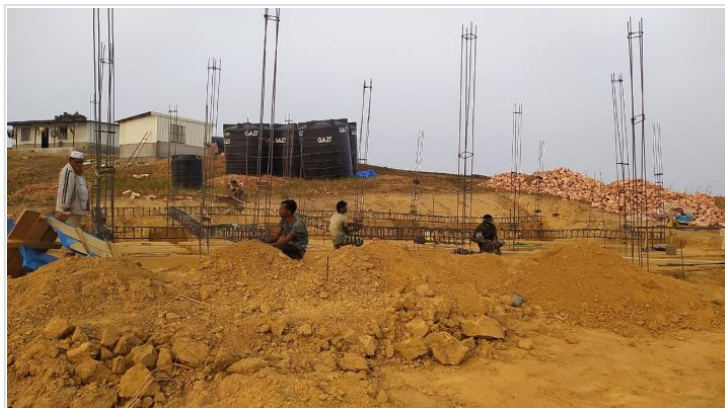
Rod binding work for grade beam at guest
