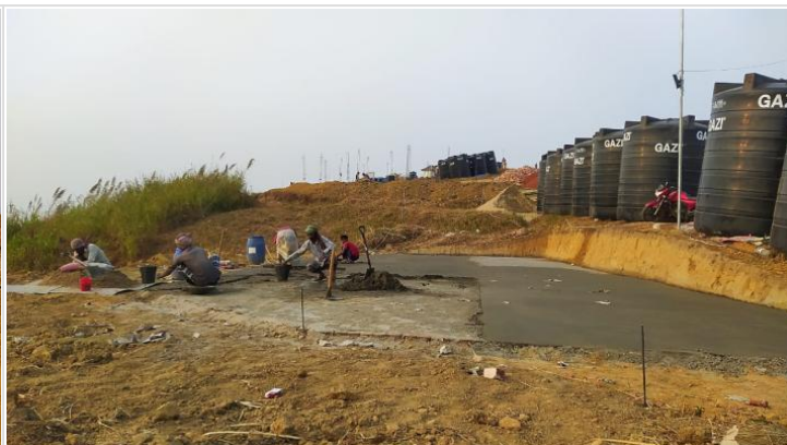
Solling joint fillup & plaster work at w
