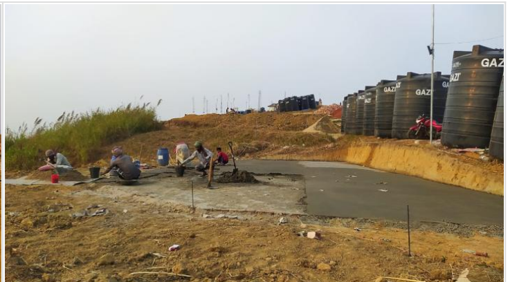
Solling joint fillup & plaster work at w
