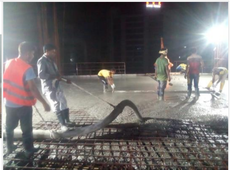
South Tower 11th Floor Slab Concreting
