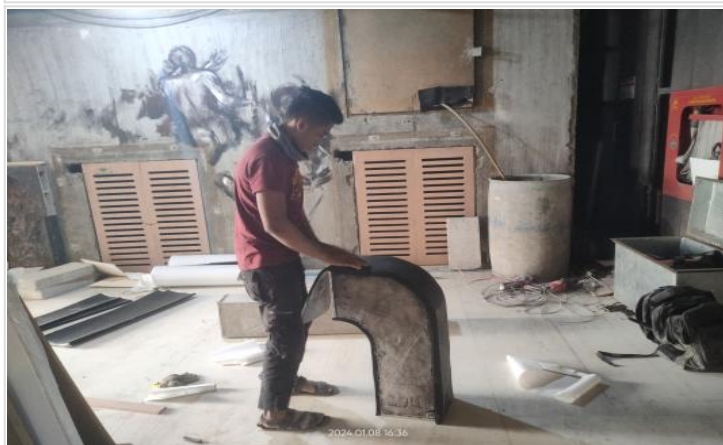
L-14-AC Duct fabrication on 08-01-24
