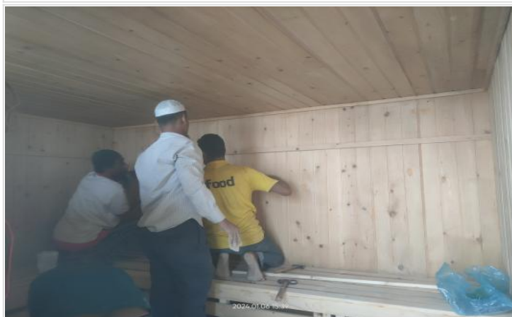
L-11-Suana-Wooden Wall Work on 06-01-24
