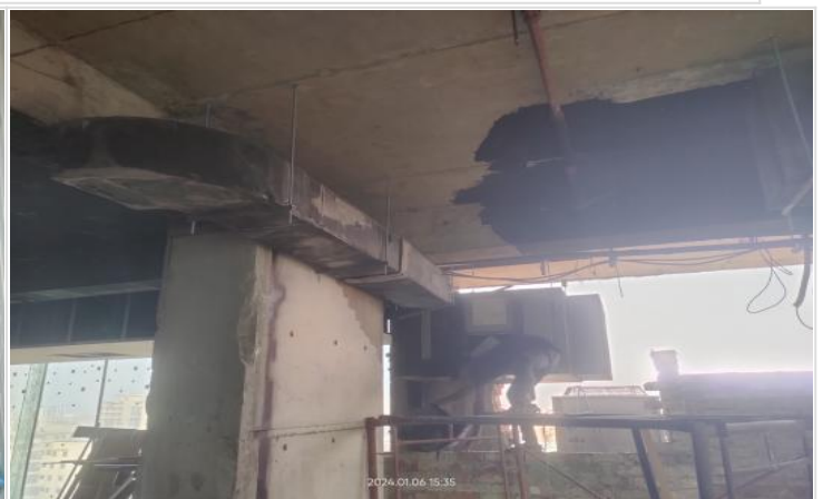
L-14-AC Duct installation on 06-01-24
