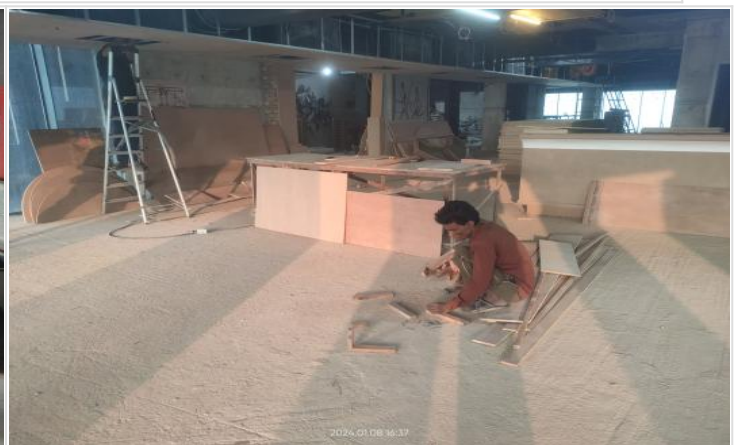
L-14-False Ceiling Work on 08-01-24
