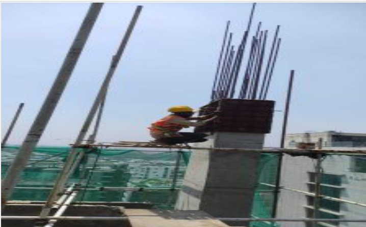
L-16-Column shuttering on 13-04-23
