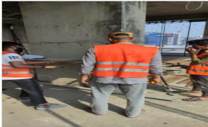
L-16-Column Stirrups making on 02-04-23
