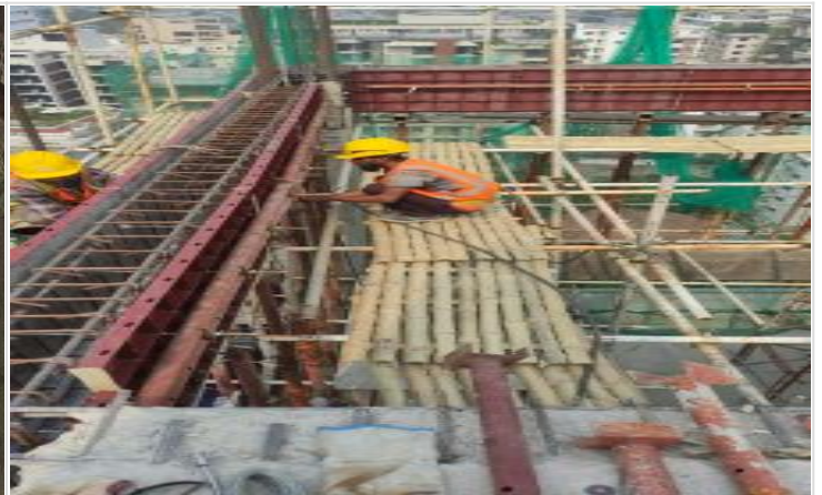
L-16-Beam shuttering on 18-04-23
