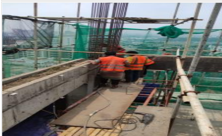
L-16-Column Re-bar on 05-04-23
