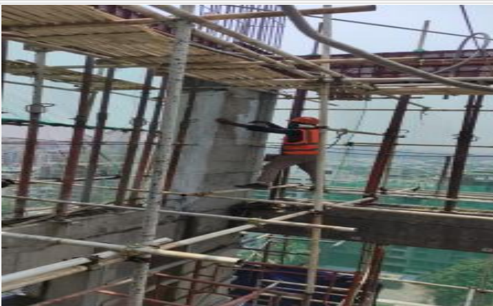
L-16-Column curing chemical applying on 19-04-23
