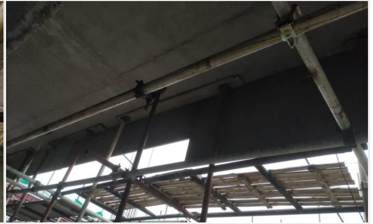
L-16-Drop Wall Shuttering on 29-04-23
