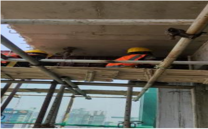
L-16-Beam Shutter removing on 29-04-23
