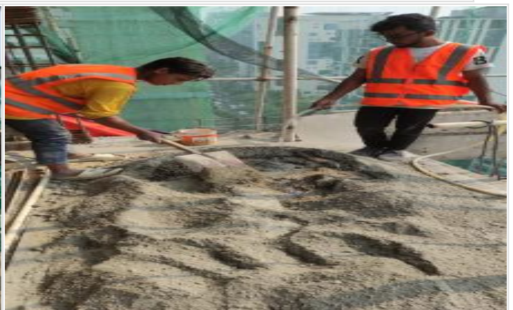
L-16-Column concrete mixing on 05-04-23
