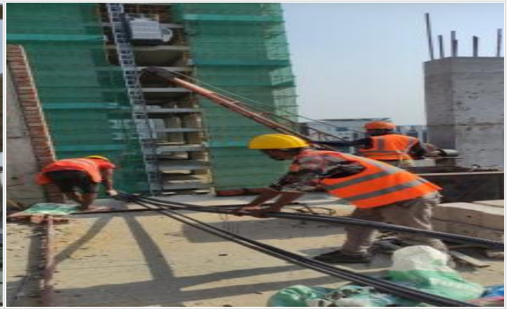
L-16-Beam Re-bar fabrication on 15-04-23
