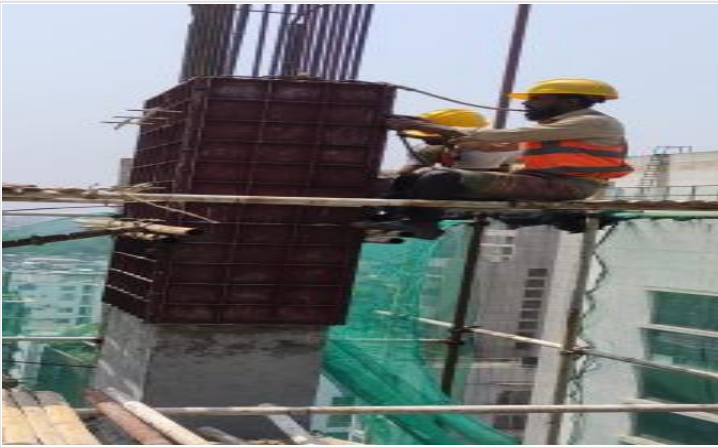
L-16-Column Shuttering on 09-04-23
