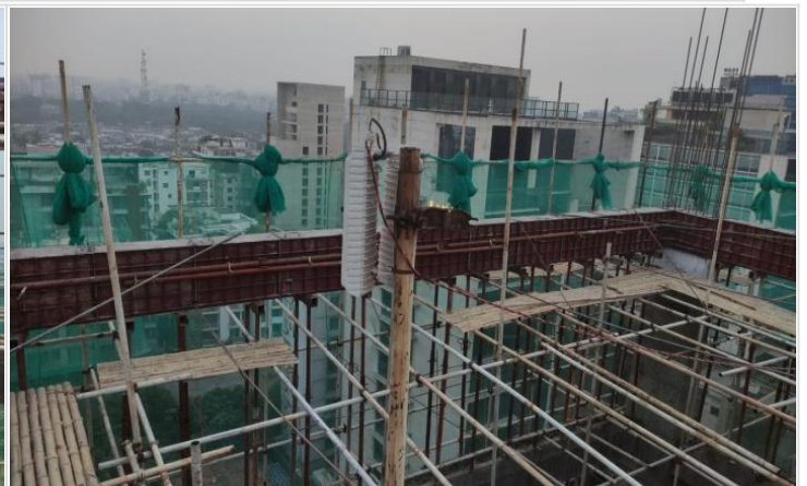
L-16-Beam concreting complete on 19-04-23
