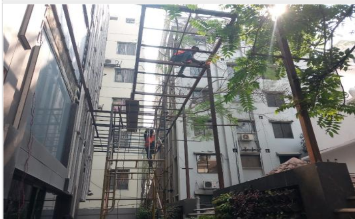
Coffee shop outside shed sheeting on 09-03-23
