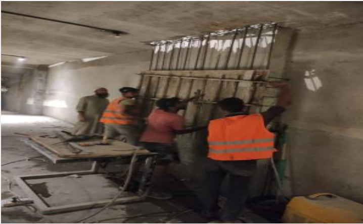
B-2-Column retrofit shuttering on 02-04-23
