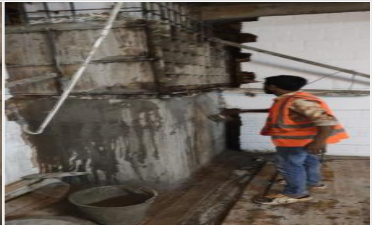
B-2-Column retrofit curing on 05-04-23
