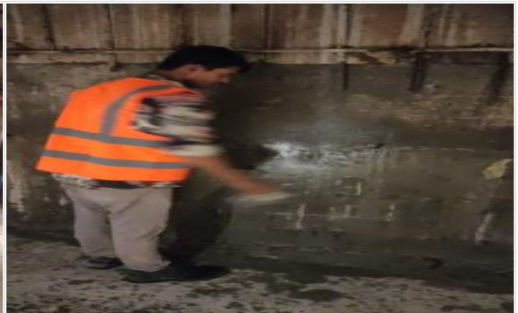
B2-Column Retrofit-Curing on 09-04-23
