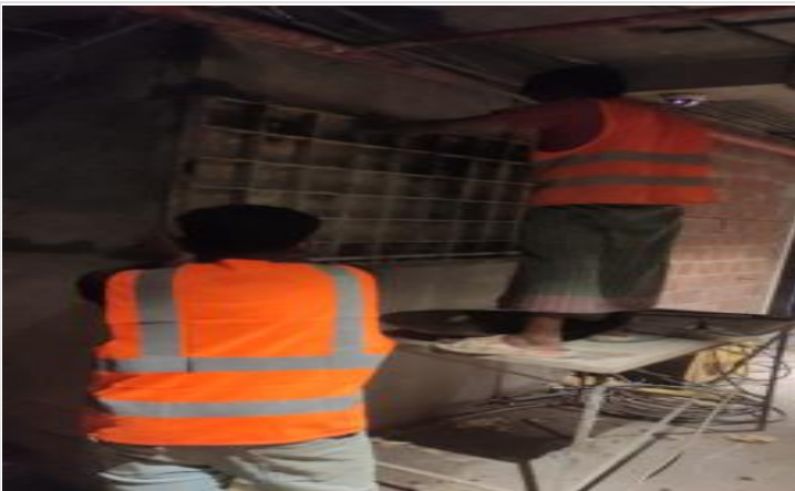
B2-Column Retrofit-Shutter removing on 09-04-23
