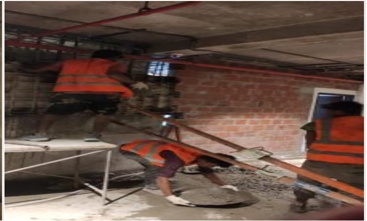
B2-Column retrofit concreting on 02-04-23
