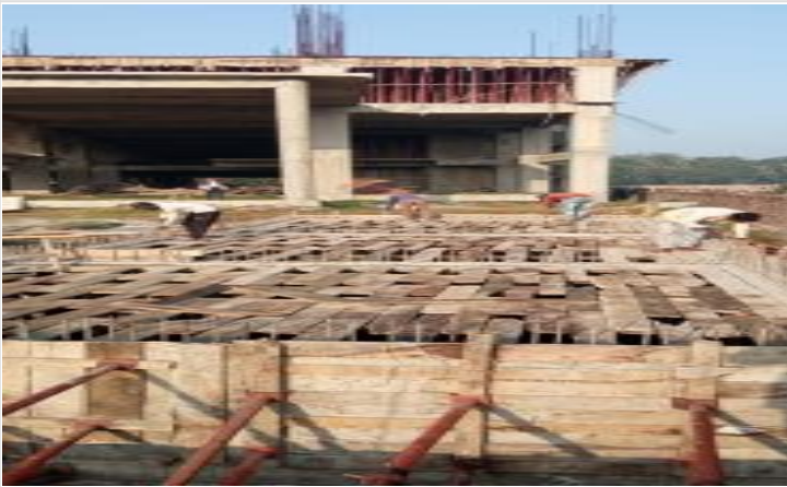
East Septic Tank Slab Shuttering on 10-02-22
