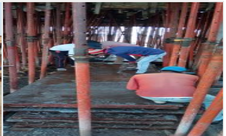
Column/Wall Steel Shutter Cleaning, Oili on 21-02-22
