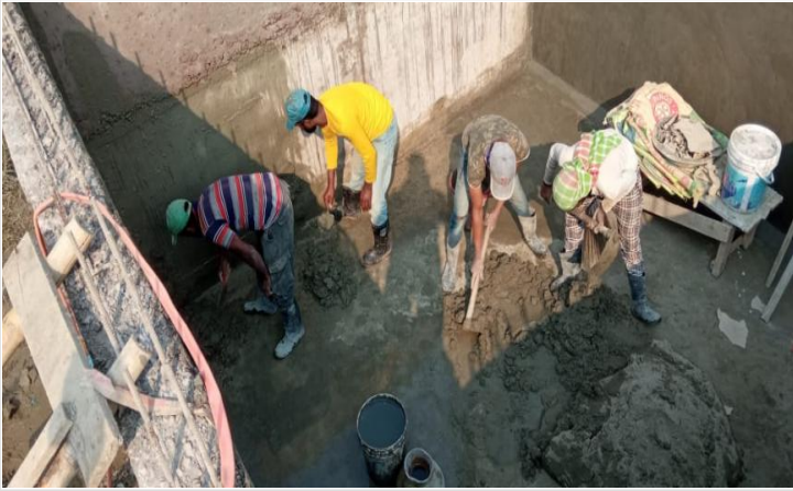
East Septic Tank Plastering on 01-02-22
