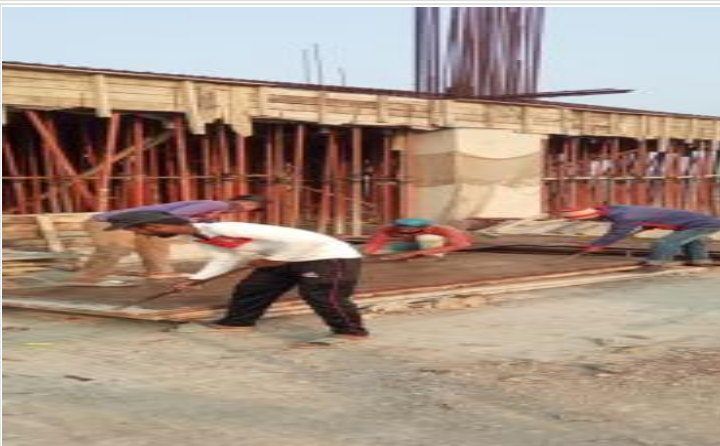
Column/Wall Steel Shutter Cleaning, Oili on 21-02-22
