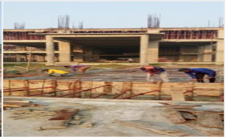
East Septic Tank Slab Shuttering on 10-02-22
