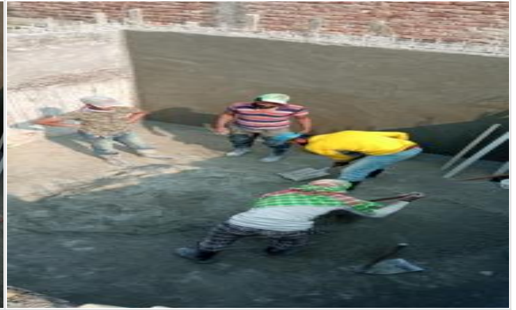
East Septic Tank Plastering on 01-02-22
