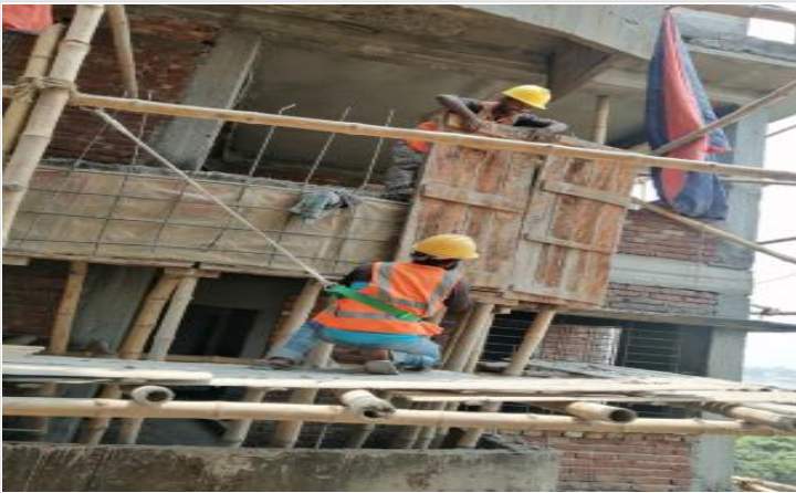
Drop Wall Shuttering on 01-05-21
