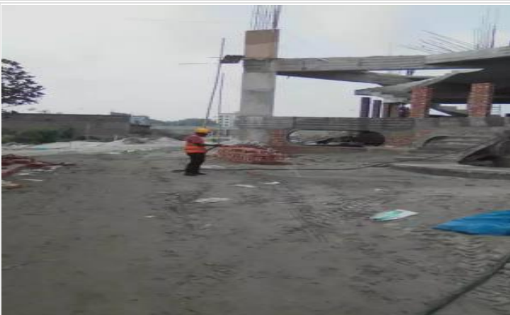
Mosque-Gr/1st Floor-Anciliary works on 04-05-21
