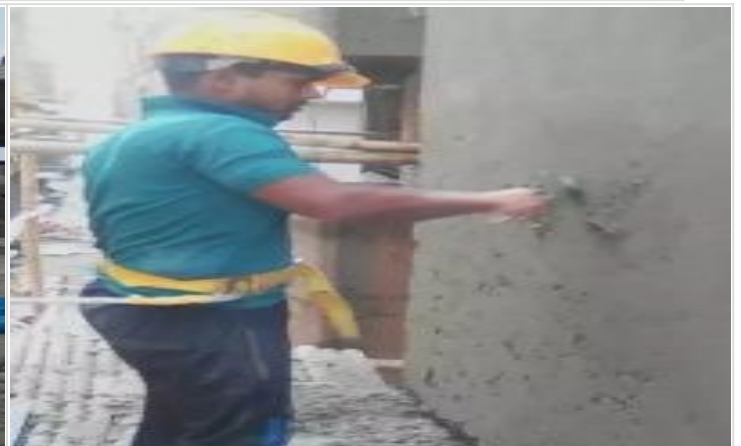
Out-side Plaster Work on 04-05-21
