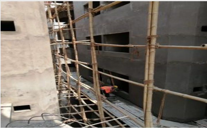
Out-side Plastering on 02-05-21
