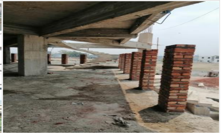
Out-side Plaster Work on 01-05-21
