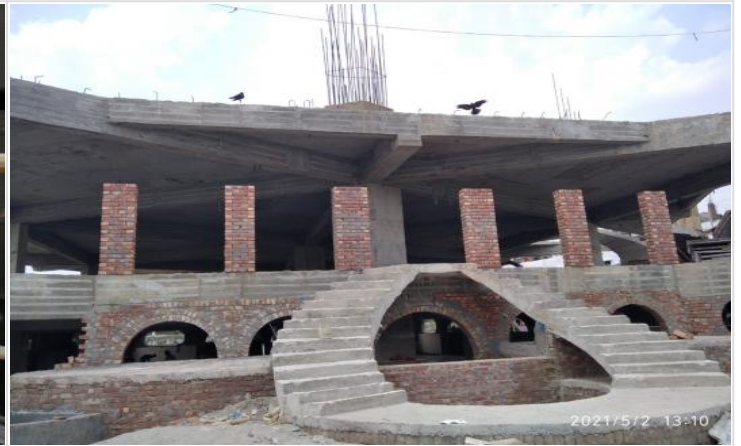
Mosque-Gr./1st Floor-Ancillary Works on 02-05-21
