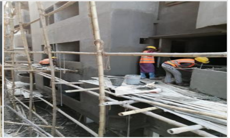
Bulding-Q-Out-side Plastering on 09-05-21
