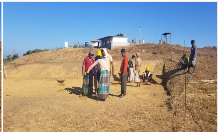
Guest House-Preparation for Layout on 07-01-21
