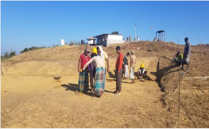
Guest House-Preparation for Layout on 05-01-21
