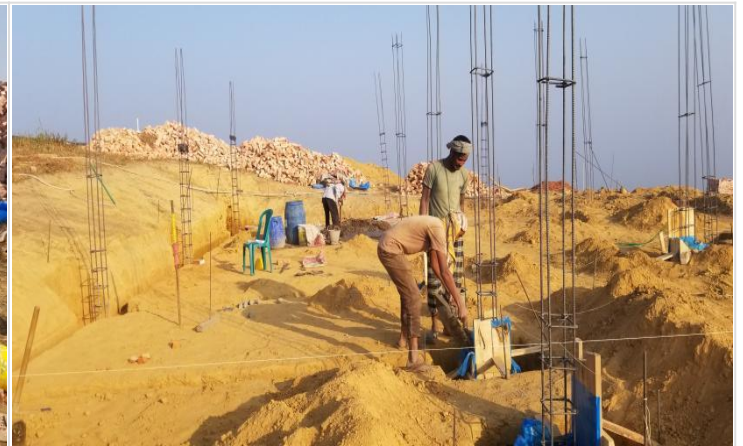
Short column casting work for guest hous on 17-01-21
