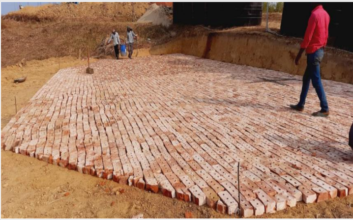
Soling for PVC Water Tank on 20-01-21
