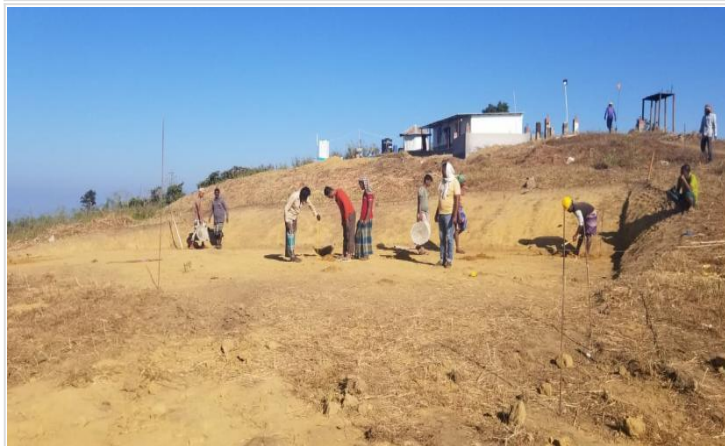
Guest House-Preparation for Layout on 07-01-21
