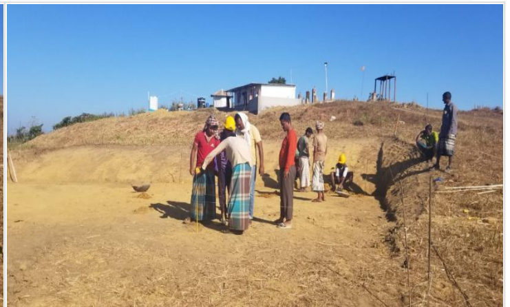
Guest House-Preparation for Layout on 06-01-21
