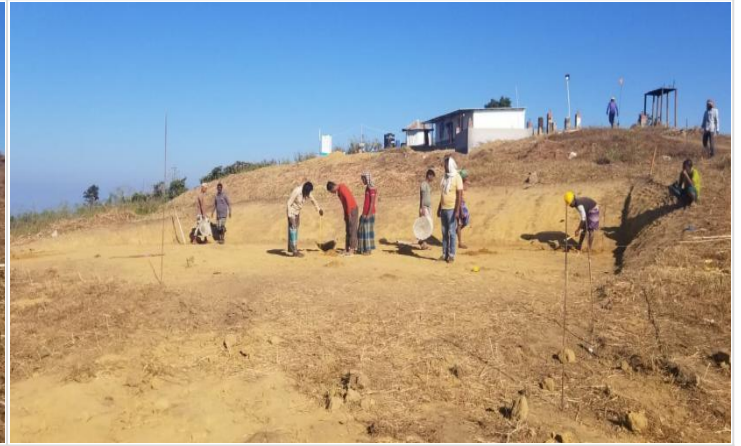
Guest House-Preparation for Layout on 05-01-21
