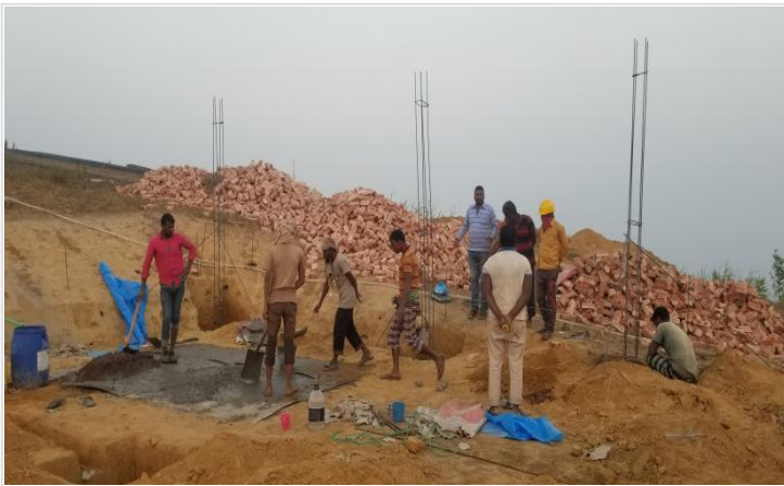
Footing & column casting work on going on 13-01-21
