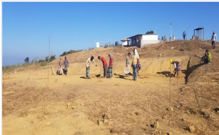
Guest House-Preparation for Layout on 06-01-21
