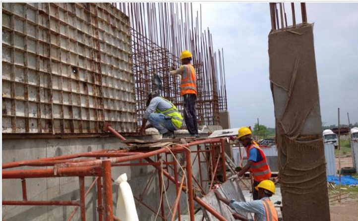
Ground Floor Lift Core Shuttering on 15-06-21
