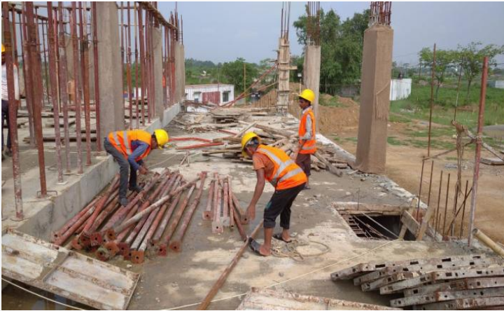
1st Floor Slab Shuttering on 03-06-21
