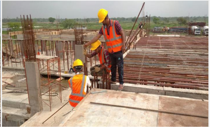
1st Floor Slab Shutter Levelling on 03-06-21
