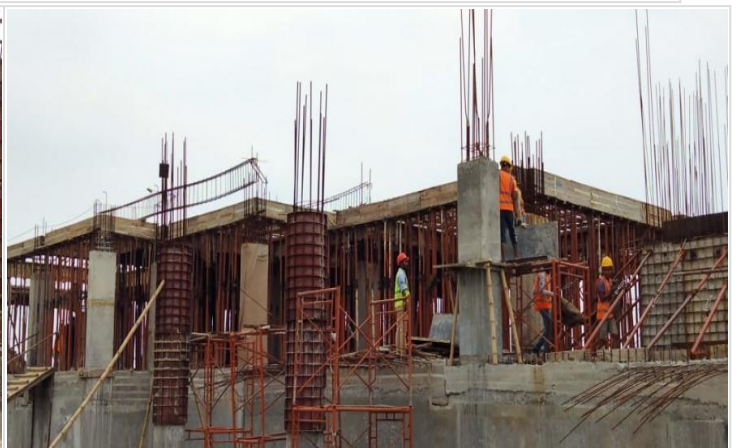
Ground Floor Construction on 07-06-21
