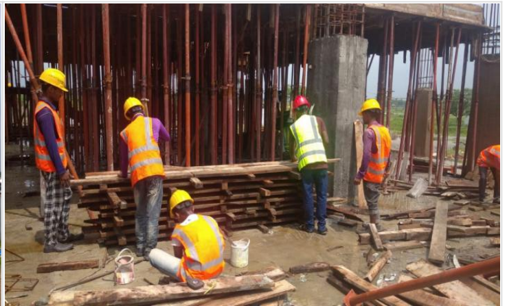
1st floor Slab Shuttering on 15-06-21
