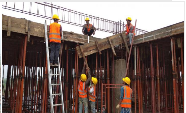
1st Floor Beam Shuttering on 06-06-21
