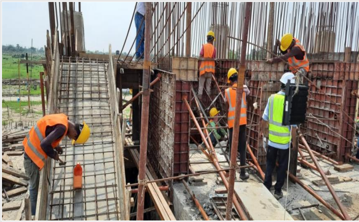
Ground Floor Stair Re-bar work on 09-06-21
