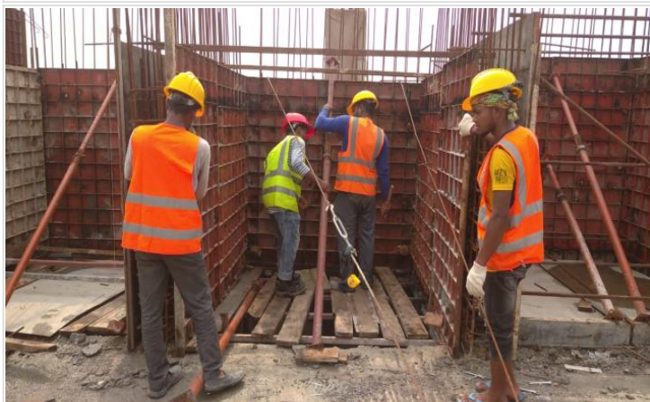
Ground floor Lift Core Shuttering on 07-06-21
