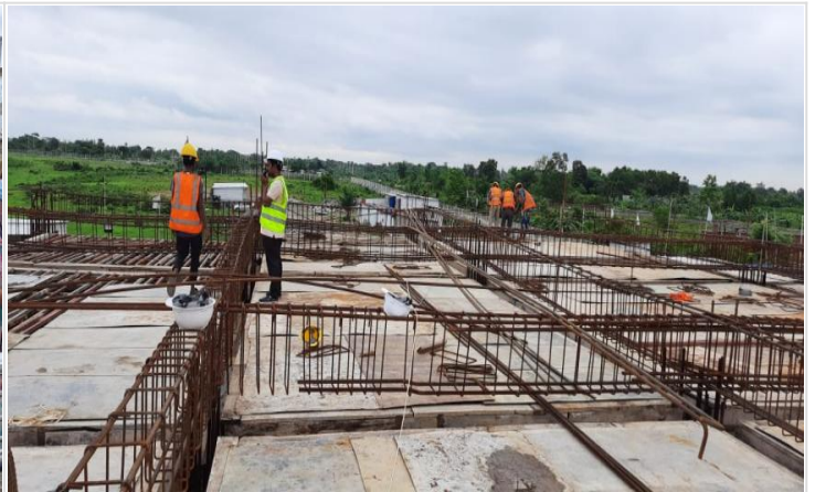
1st floor Slab Shuttering on 12-06-21
