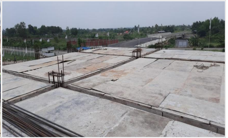
1st floor Slab Shuttering on 09-06-21
