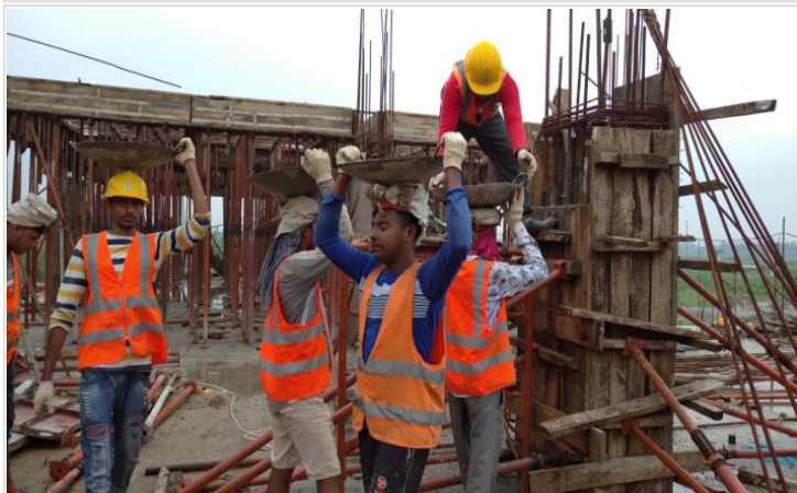
Ground Floor Column Concreting on 06-06-21
