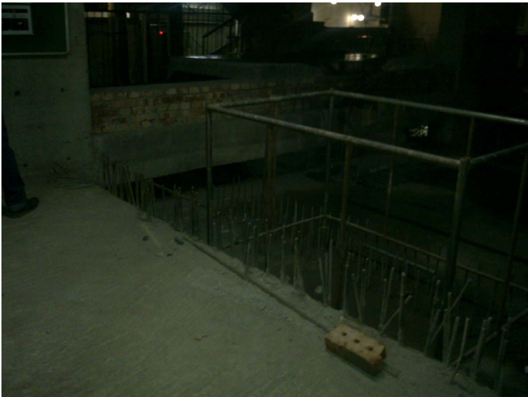
In-front of Site Office Safety Railing should be provided
