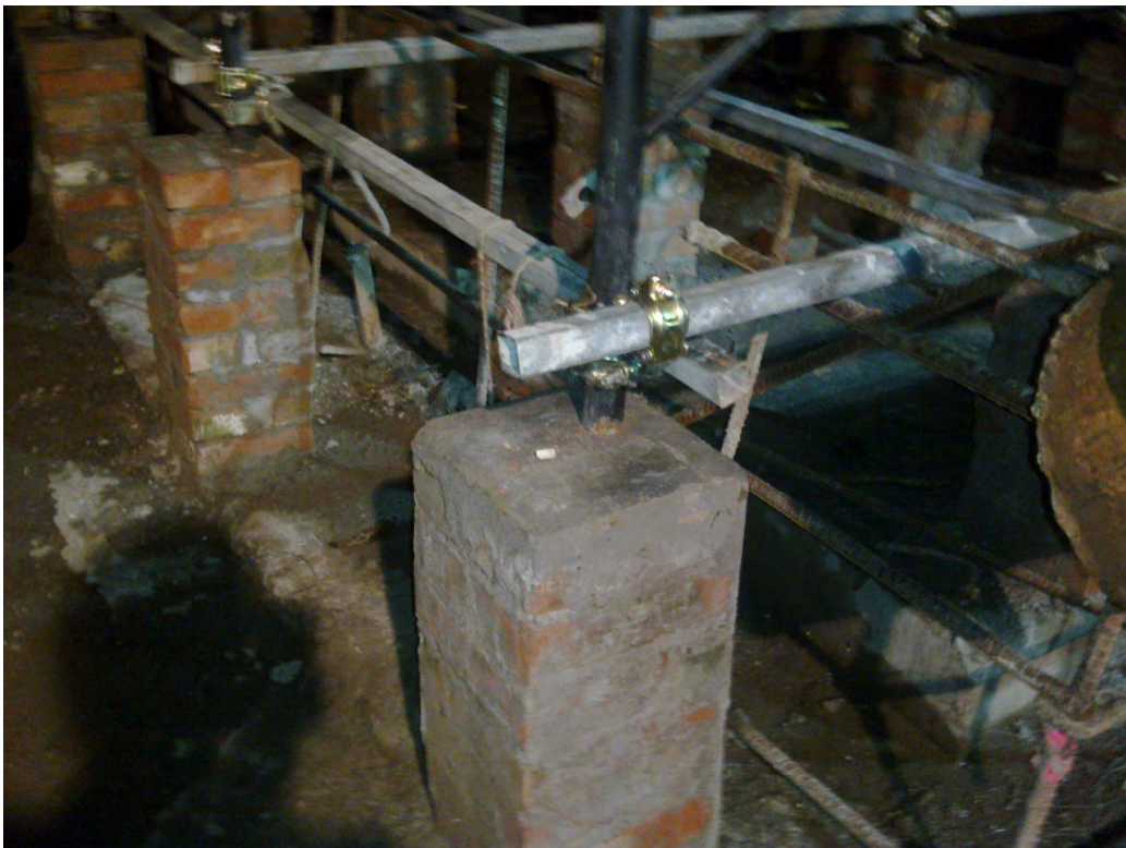
IMPROPER SCAFFOLDING-BASE PLATE NEEDED
