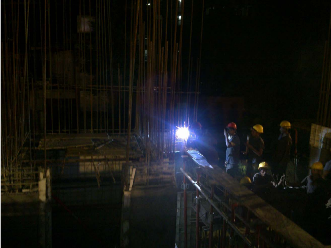
WELDING WITHOUT EYE PROTECTION(SAFETY GOGGLES) – Cause Eye Damage
