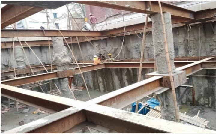
Water proofing work on 30-04-22
