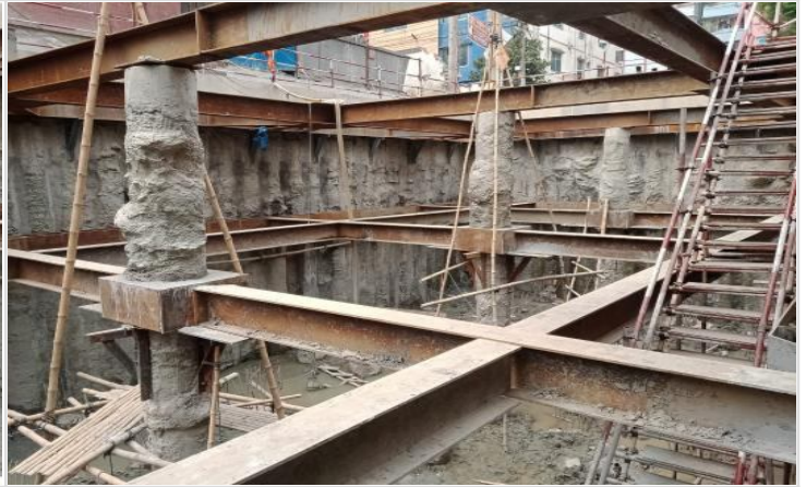
Pile gap water proofing on 30-04-22
