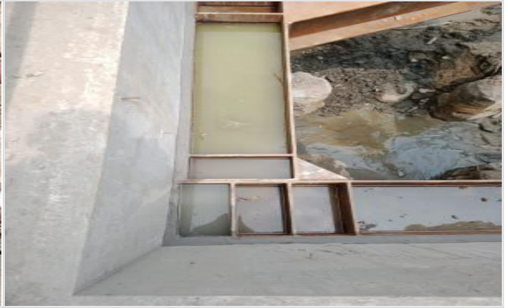
Gap filling by mortering on 02-04-22
