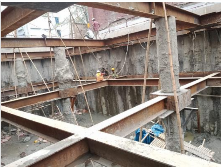
Water proofing work
