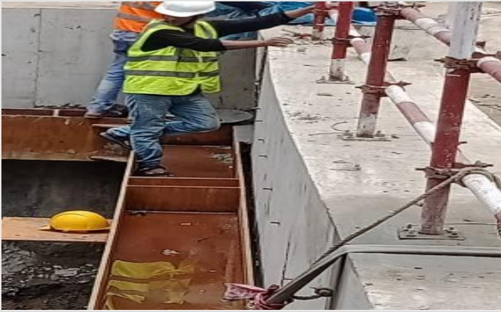
Gap filling inbetween joist and cap beam on 02-04-22
