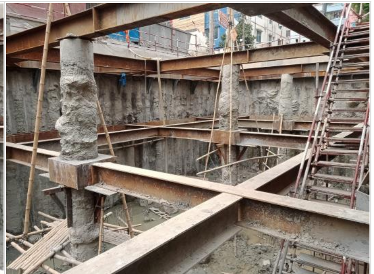
Pile gap water proofing
