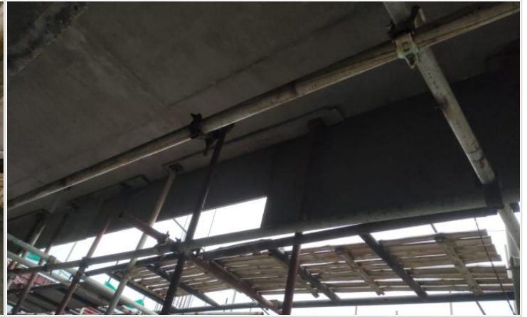
L-16-Drop Wall Shuttering on 29-04-23
