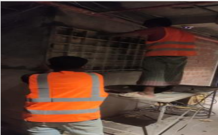
B2-Column Retrofit-Shutter removing on 09-04-23
