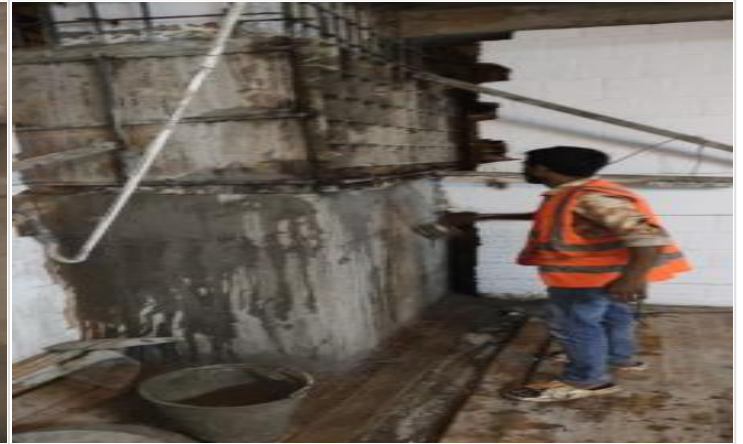
B-2-Column retrofit curing on 05-04-23
