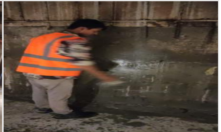
B2-Column Retrofit-Curing on 09-04-23
