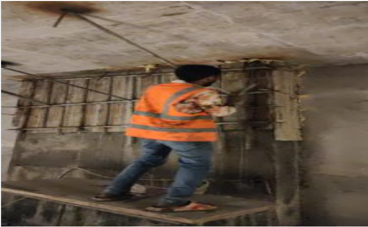
B2-Column retrofit shutter removing on 05-04-23
