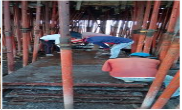
Column/Wall Steel Shutter Cleaning, Oili on 21-02-22
